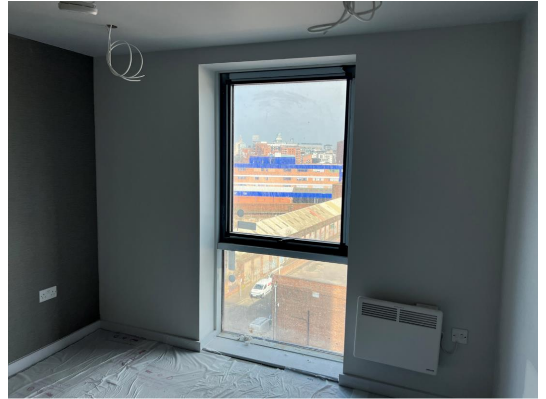
Bedroom 2 nd fix lighting
