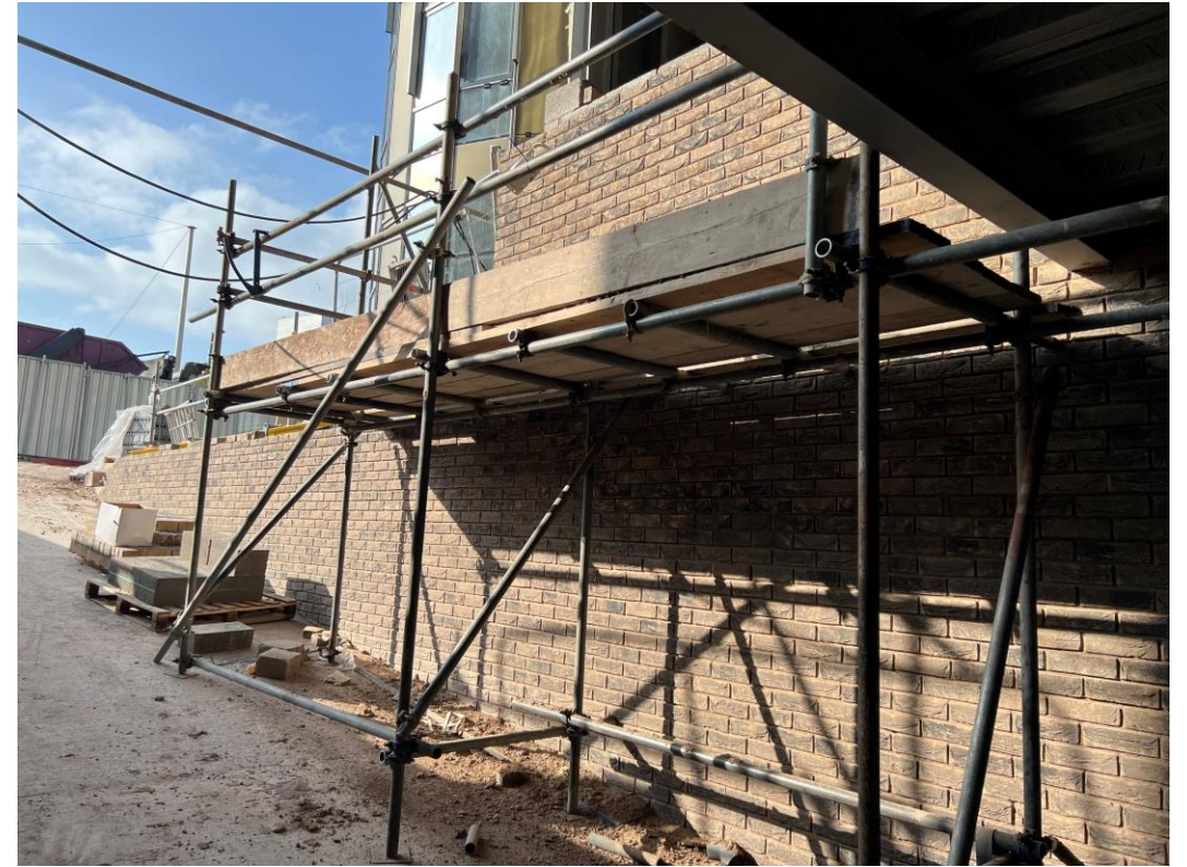
Temporary working platform for brickwork installation
