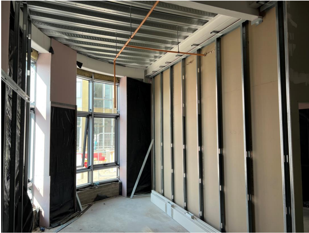
Ground Floor - Apartment construction commenced
