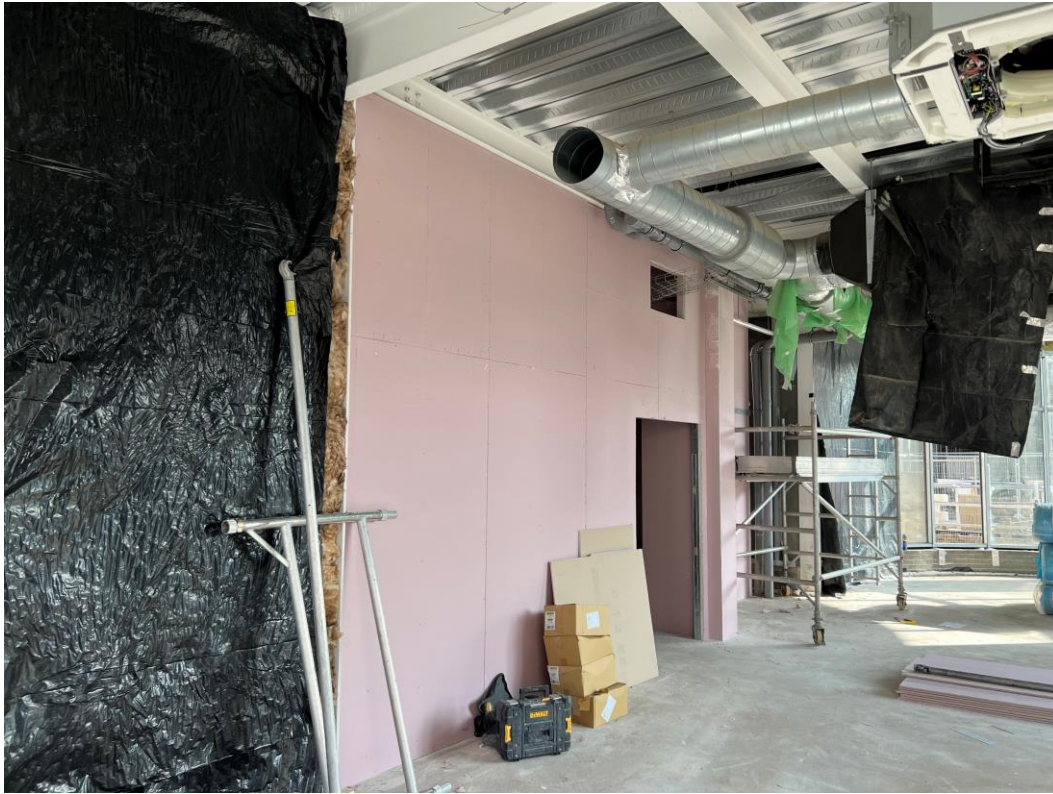
Ground Floor - Partitions installed & boarded one side
