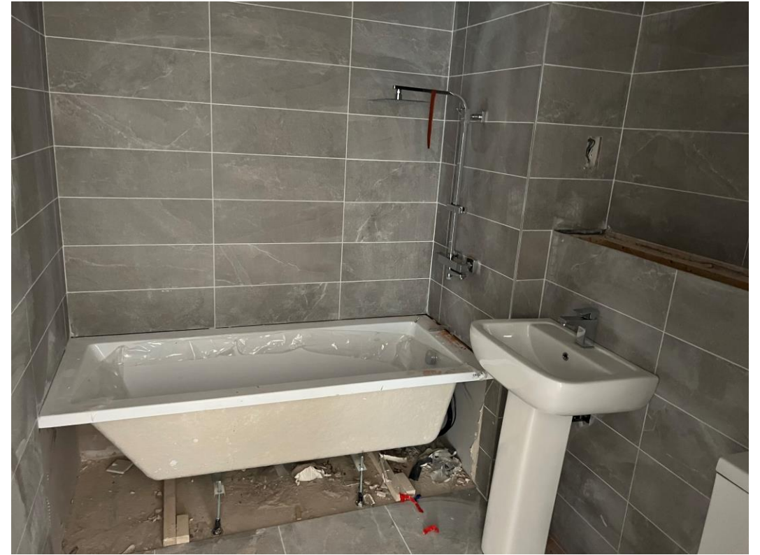
Bathroom sanitary items installed
