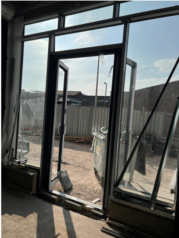
Ground Floor - Entrance doors installed
