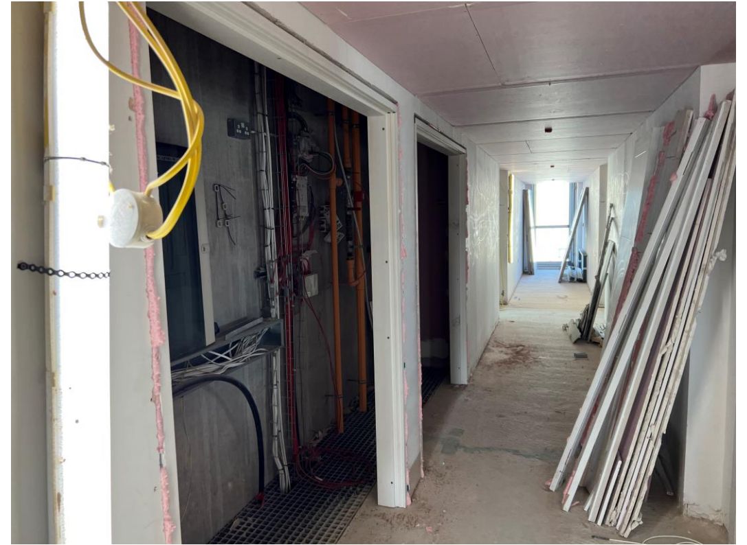
Doorframes installed
