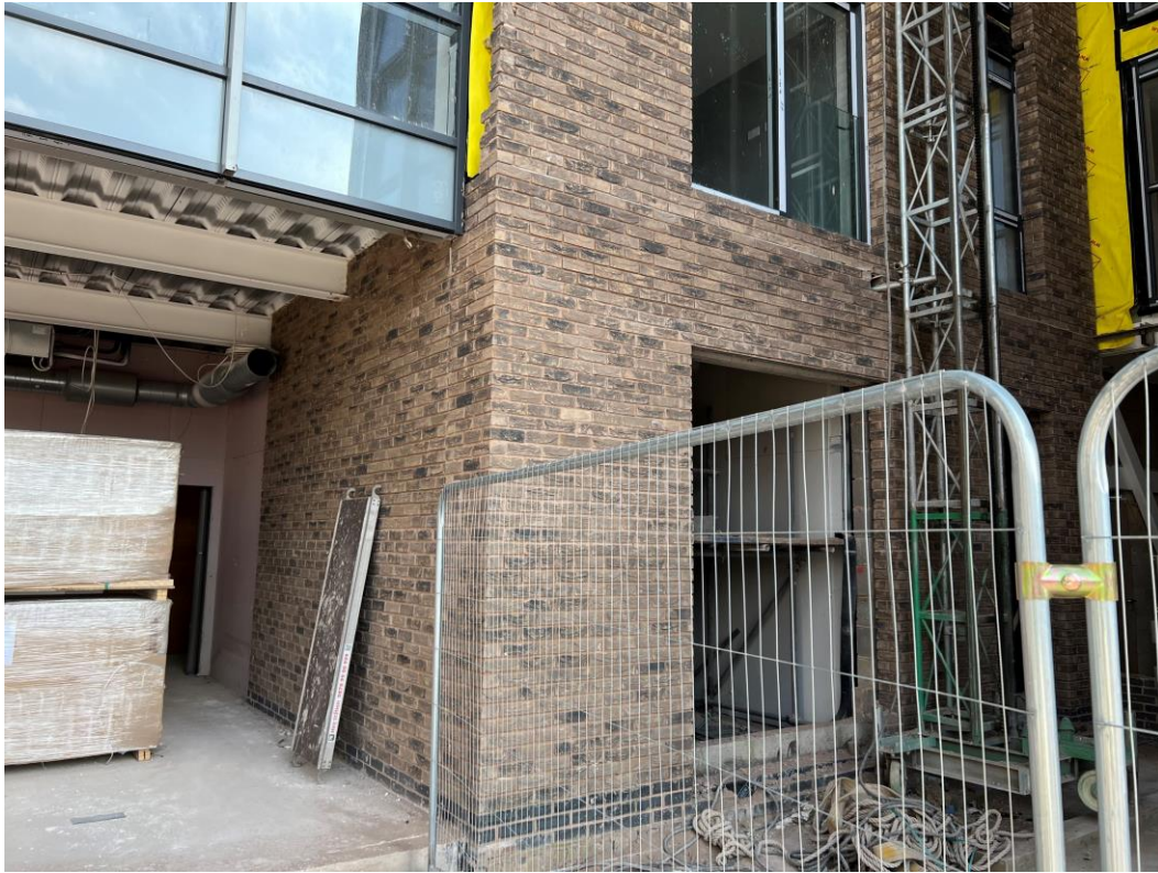
Brindley Street - External brickwork
