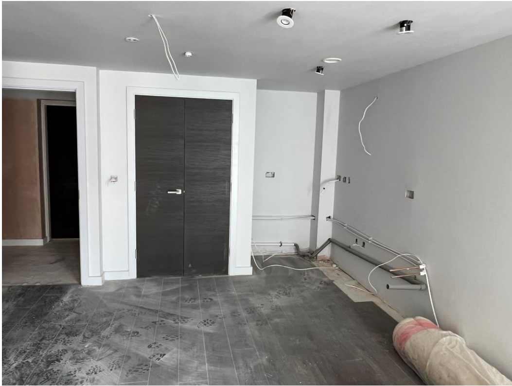
Kitchen 2 nd fix lighting installed
