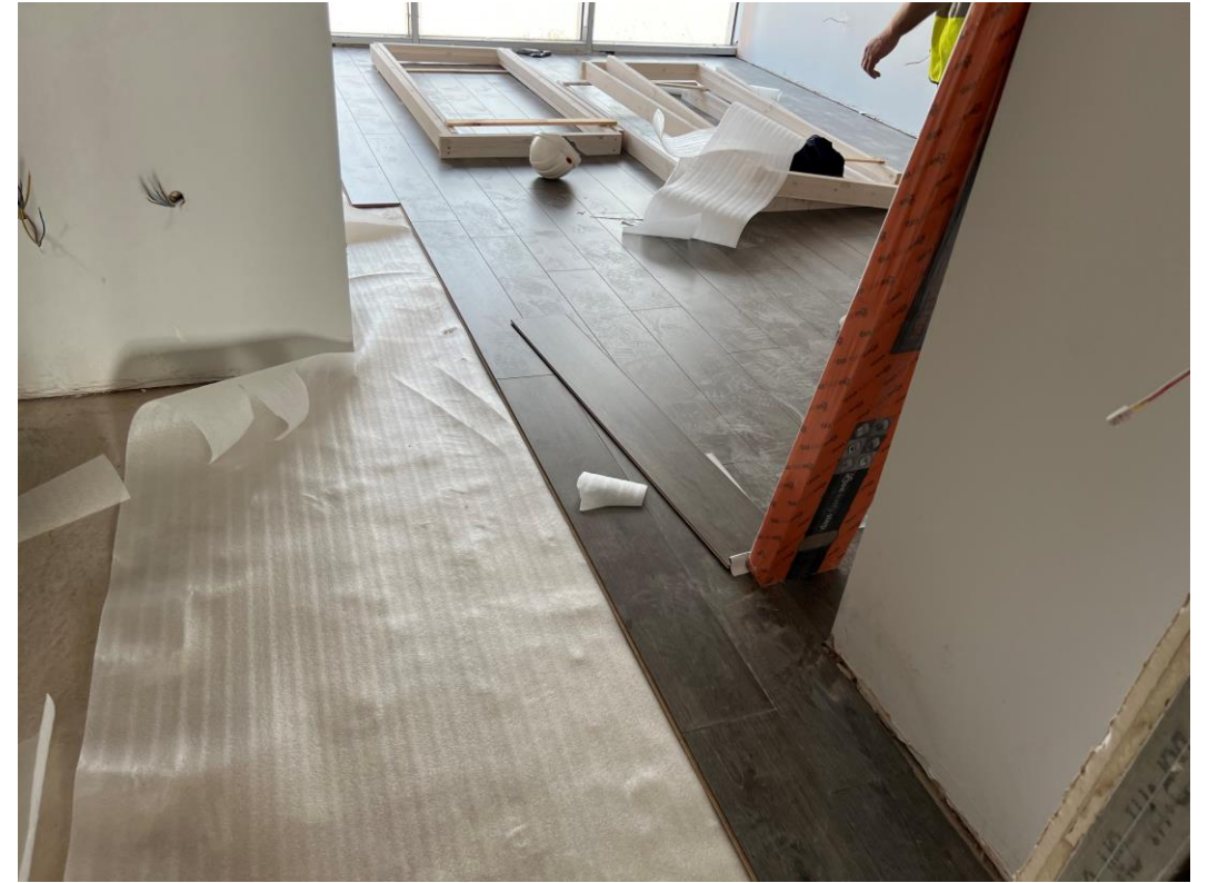
Laminate flooring installation ongoing
