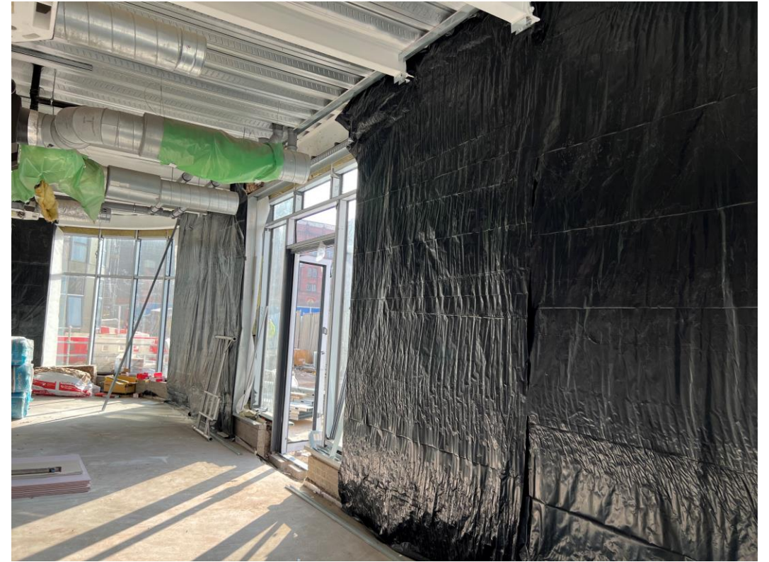
Ground Floor - VCL installed
