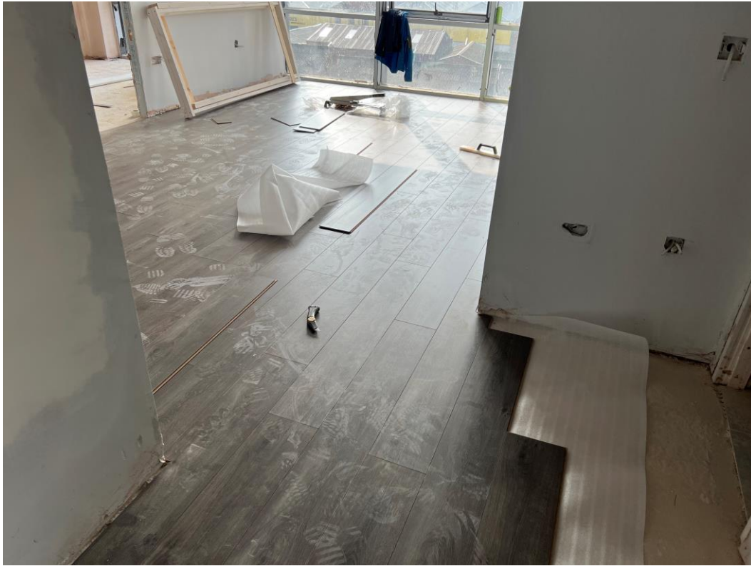
Laminate flooring installation ongoing
