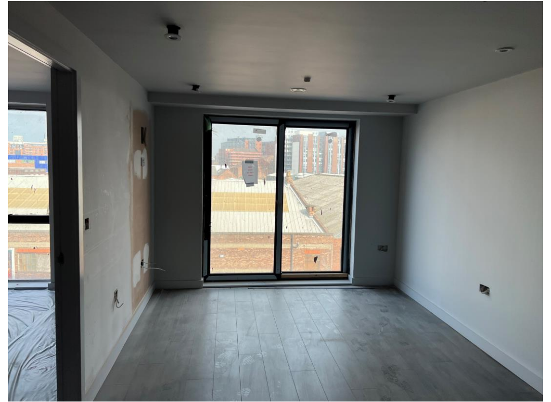
Kitchen / Lounge 2 nd fix lighting installed
