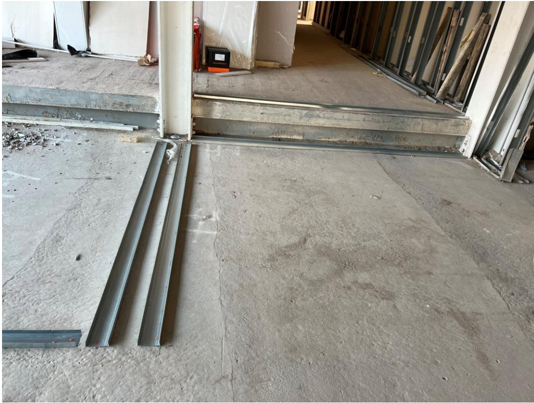
Setting out partitions
