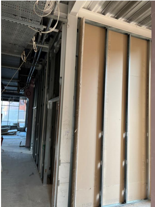
Ground Floor - Partitions installed & boarded one side
