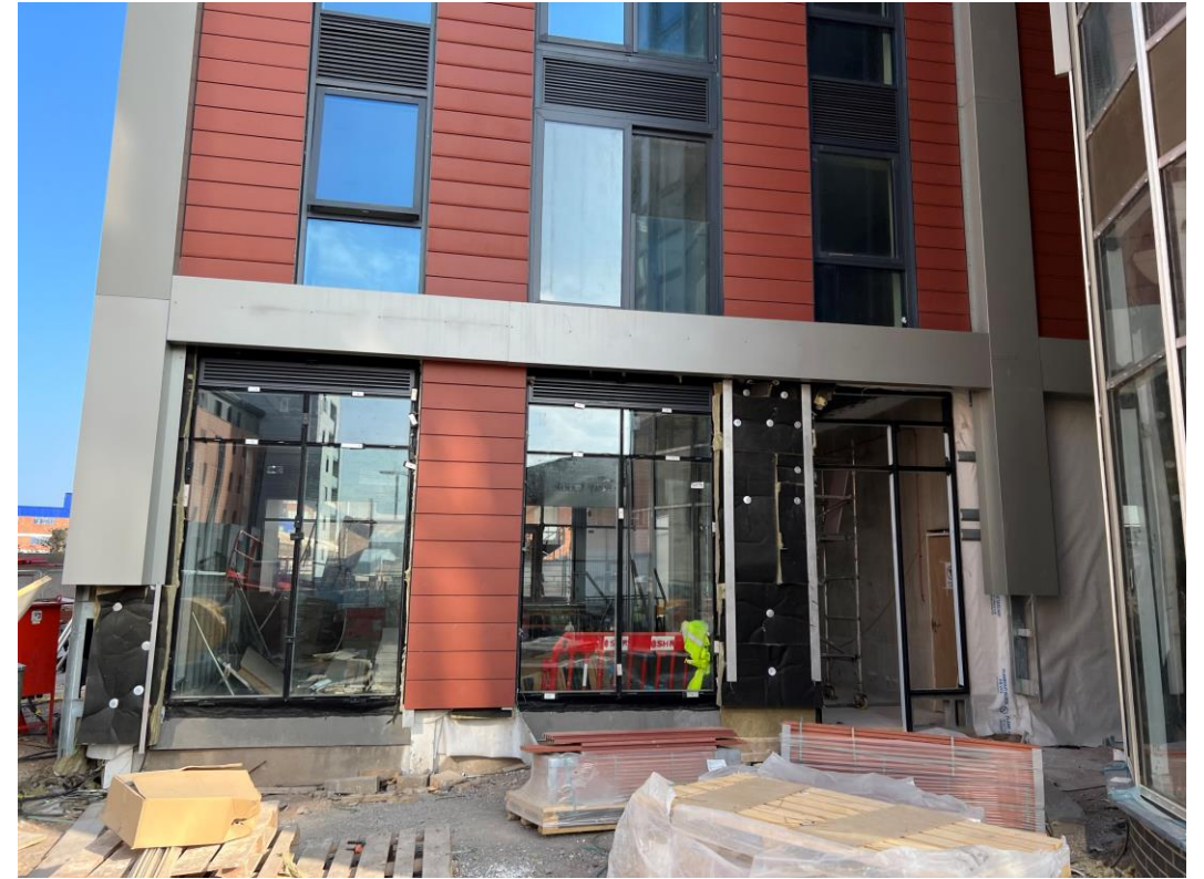
External cladding remedial works
