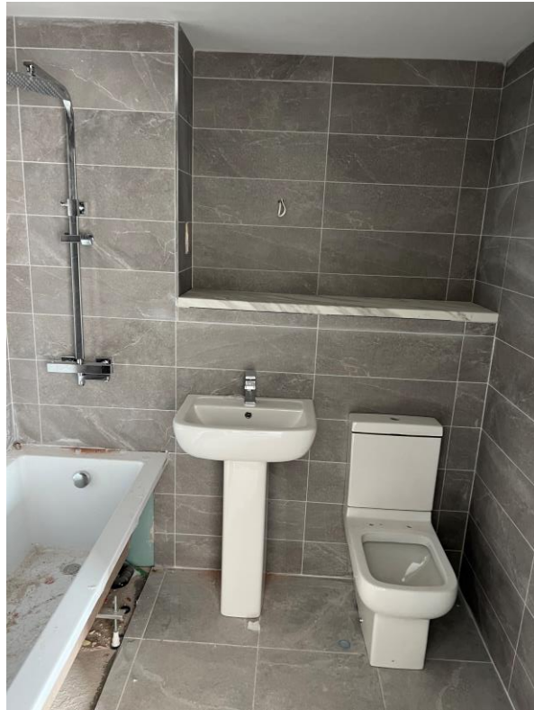
Bathroom sanitary items installed
