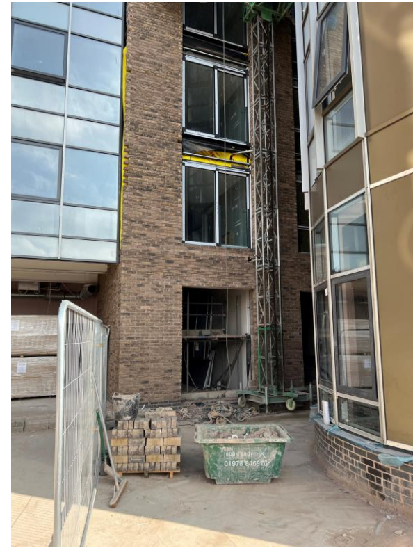
Brindley Street - External brickwork
