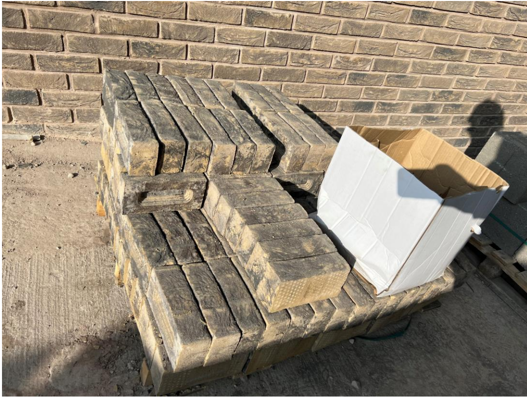
Bricks on site for installation
