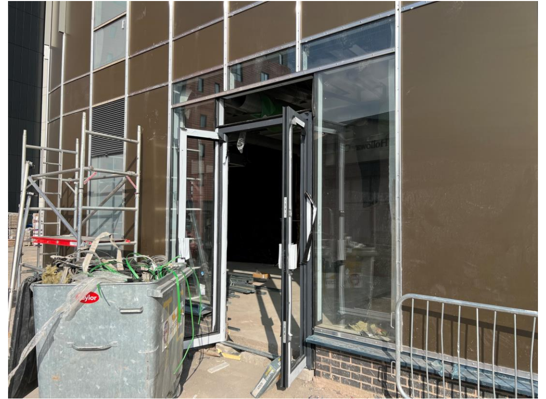
Ground Floor entrance doors installed
