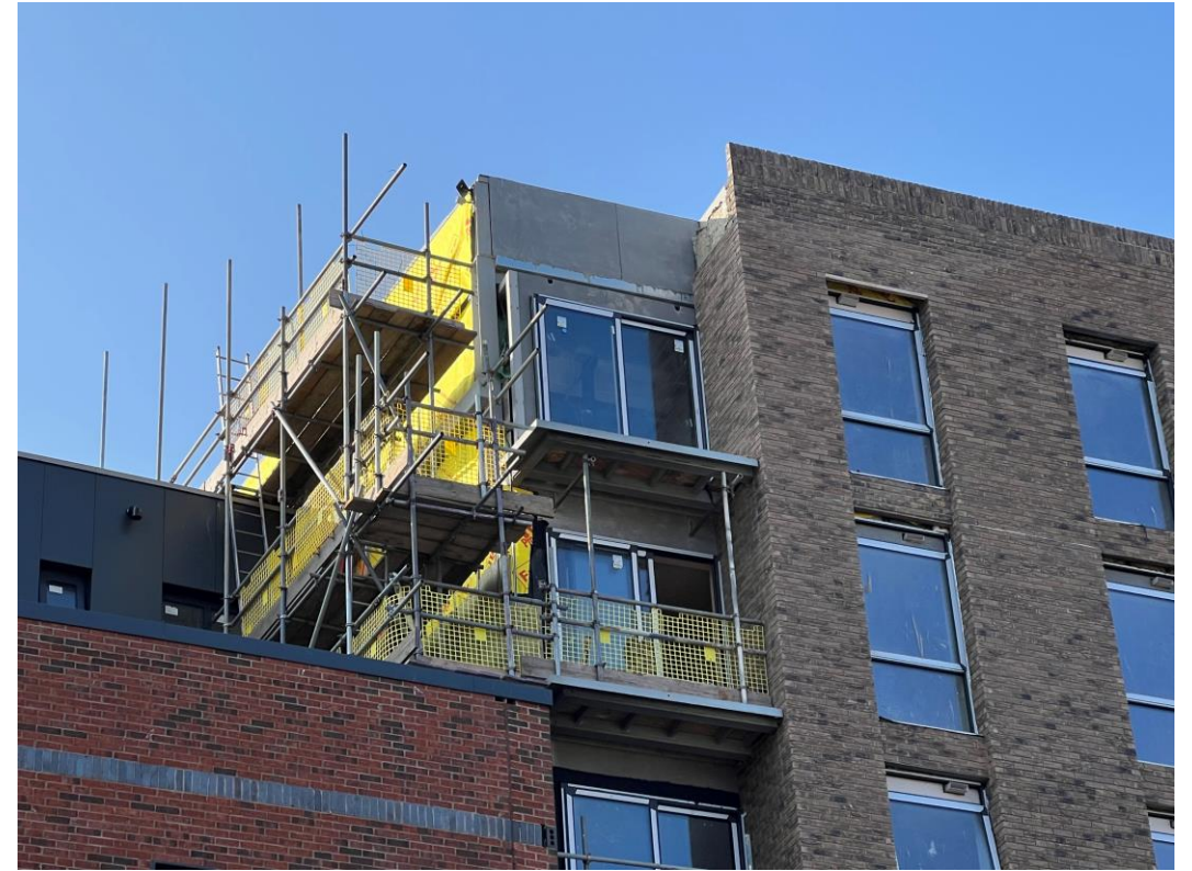
External cladding remedial works
