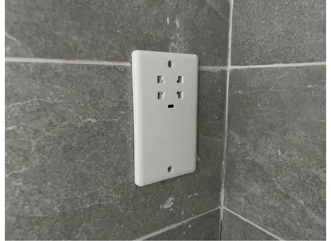
Shaving socket installed
