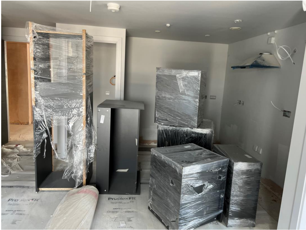
Kitchen units onsite for installation
