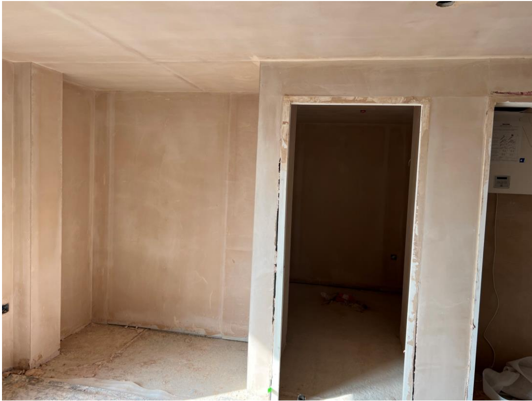
Apartment walls & ceilings plaster skimmed
