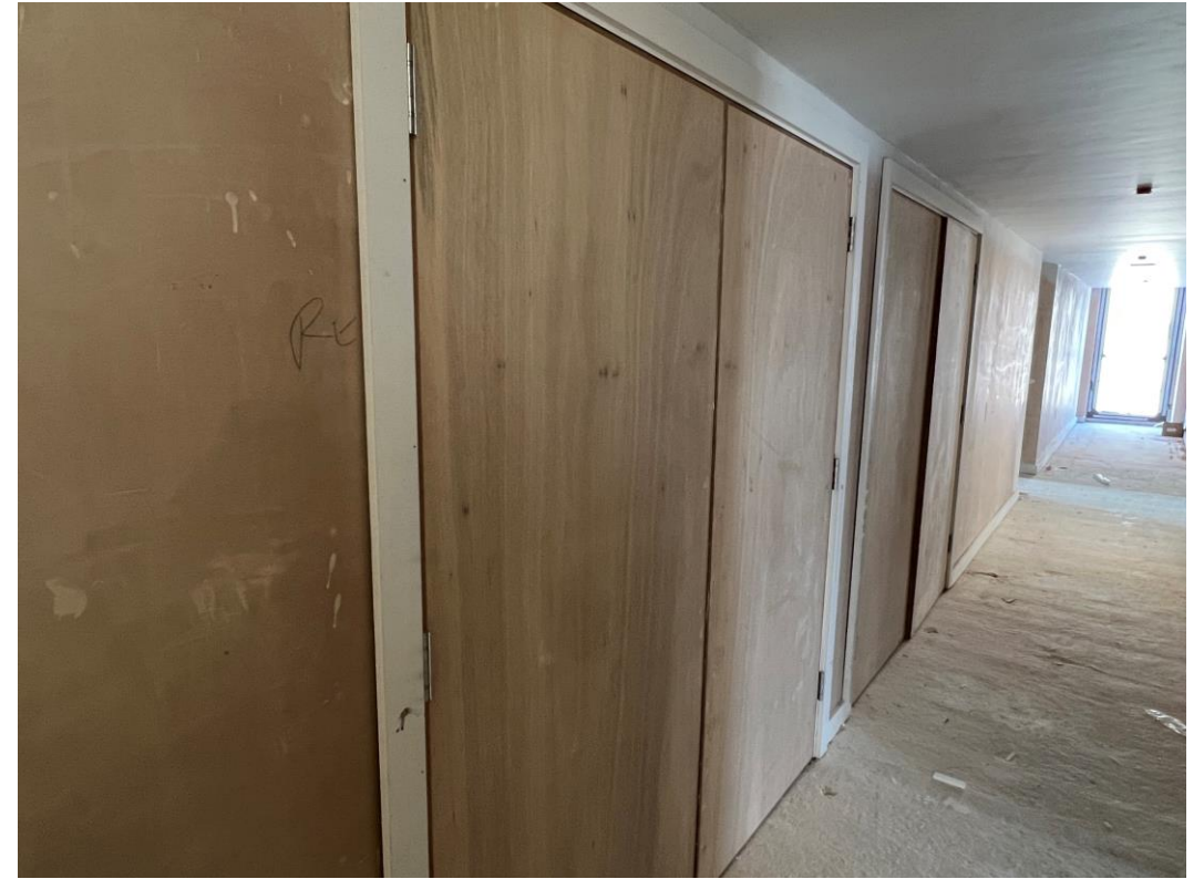
Fire doors installed
