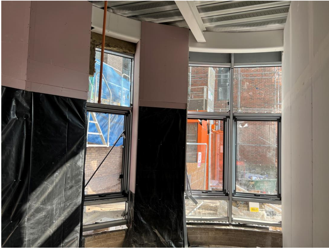
Ground Floor - Apartment construction commenced
