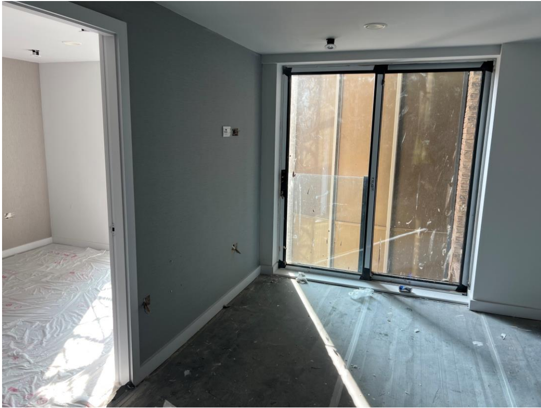
Kitchen / Lounge Finishes
