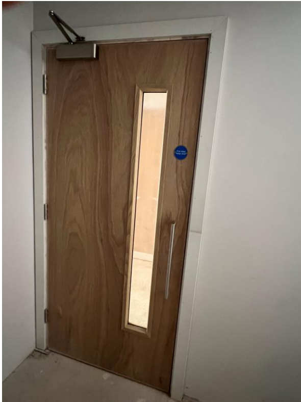
Fire door installed to staircase landing area
