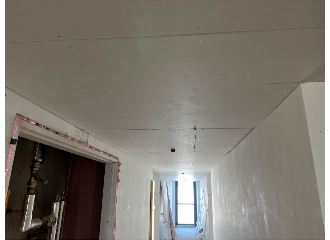
Ceilings boarded to circulation areas
