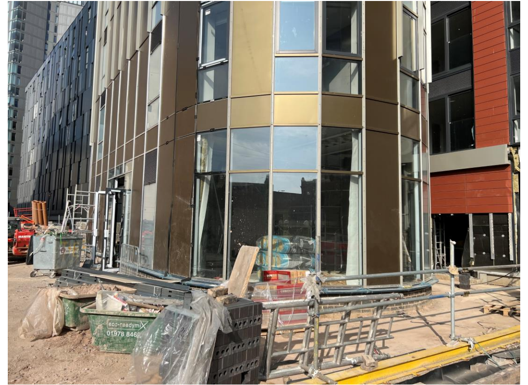
Ground Floor curtain walling
