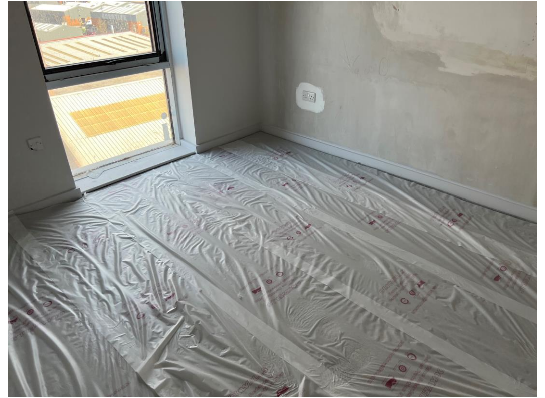
Carpets installed & protected
