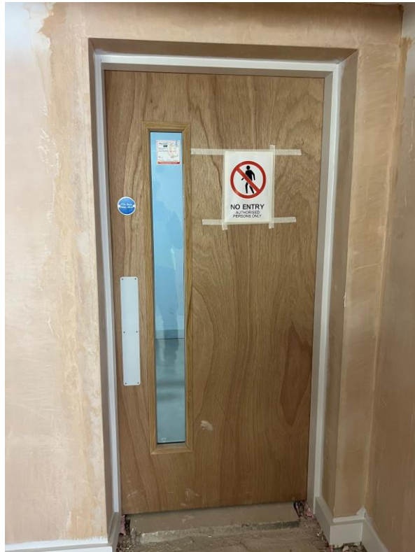
Fire door installed to staircase landing area
