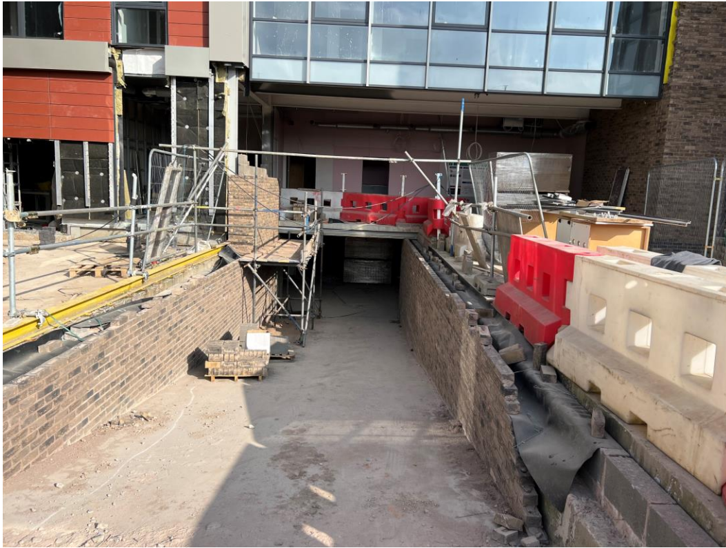
External brickwork installed to basement ramp
