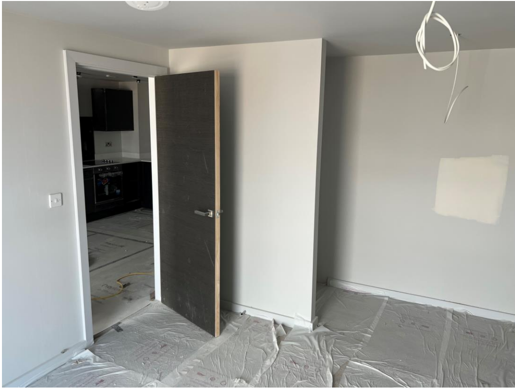
Bedroom walls and ceilings decorated
