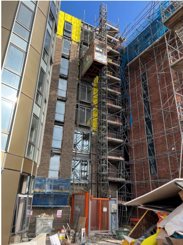
Brindley Street - External brickwork
