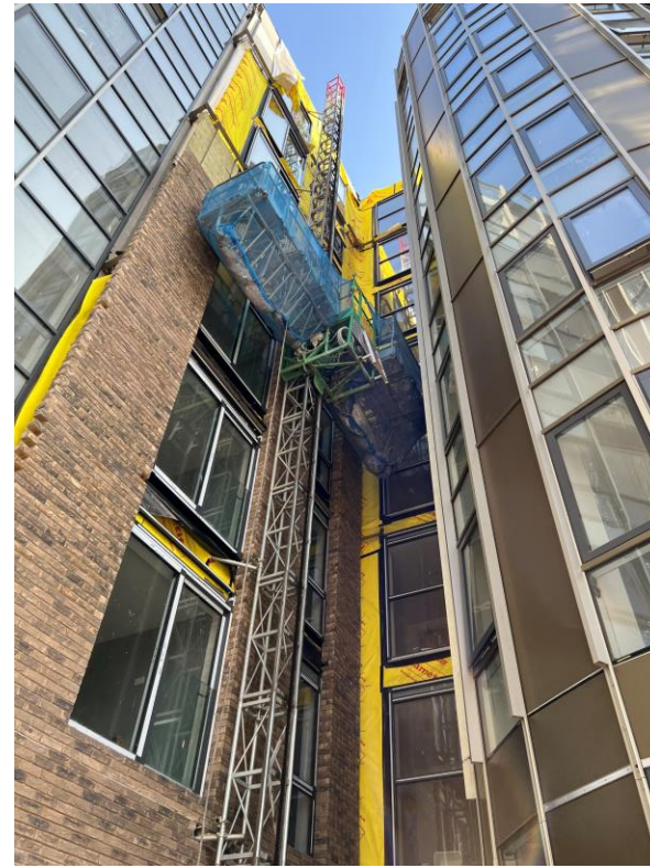
Brindley Street - External brickwork
