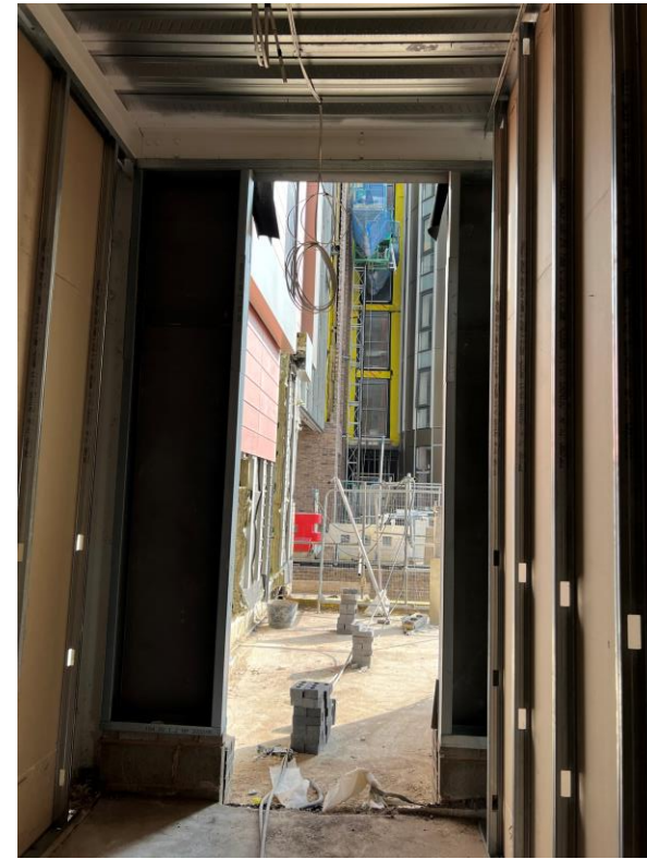
Ground Floor - Partitions installed & boarded one side
