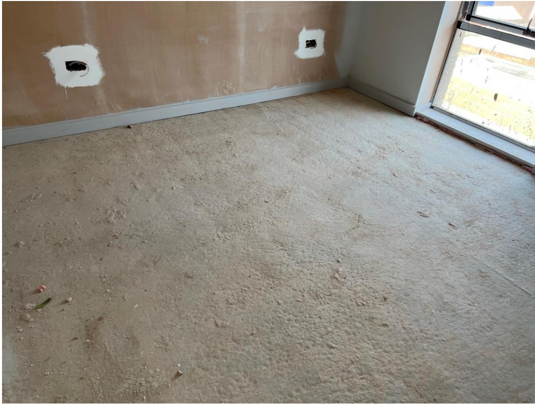
Bedroom awaiting carpet installation
