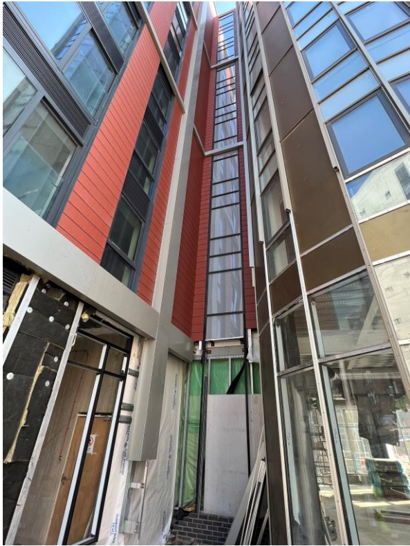
External cladding remedial works
