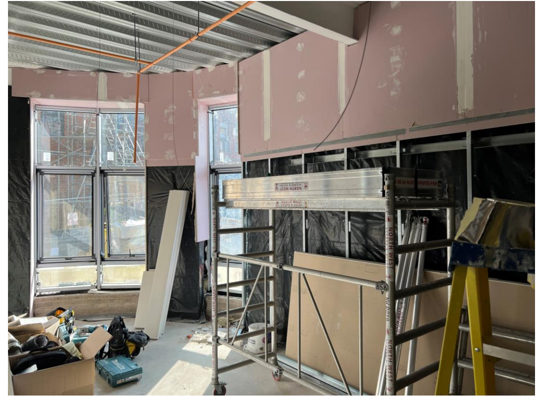
Ground Floor - Apartment construction commenced
