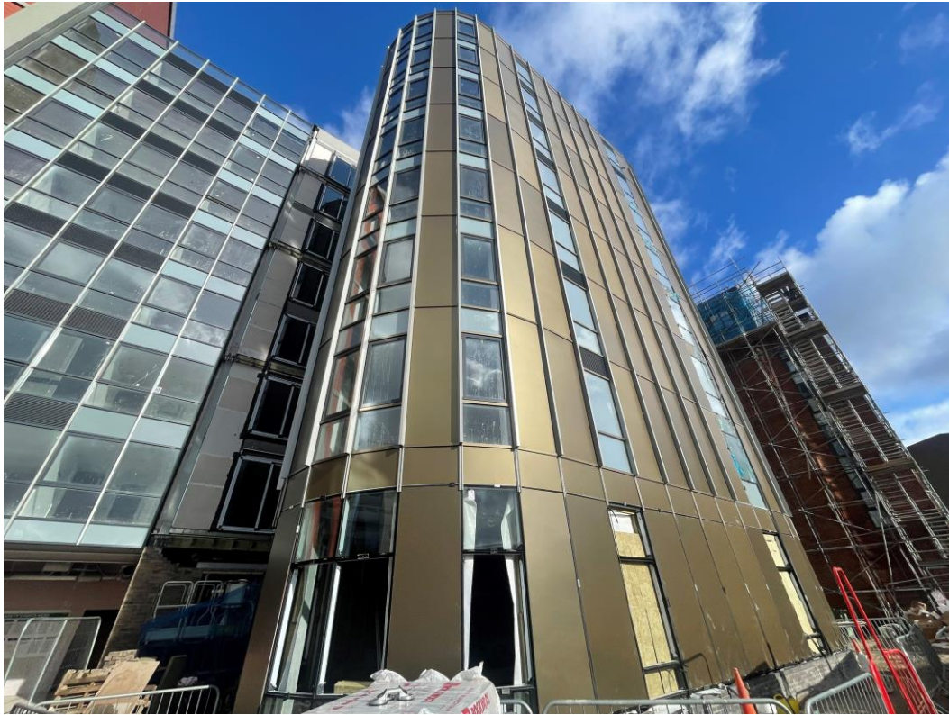
Window & glazing installation ongoing
