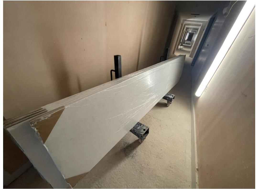
Worktops loaded for installation
