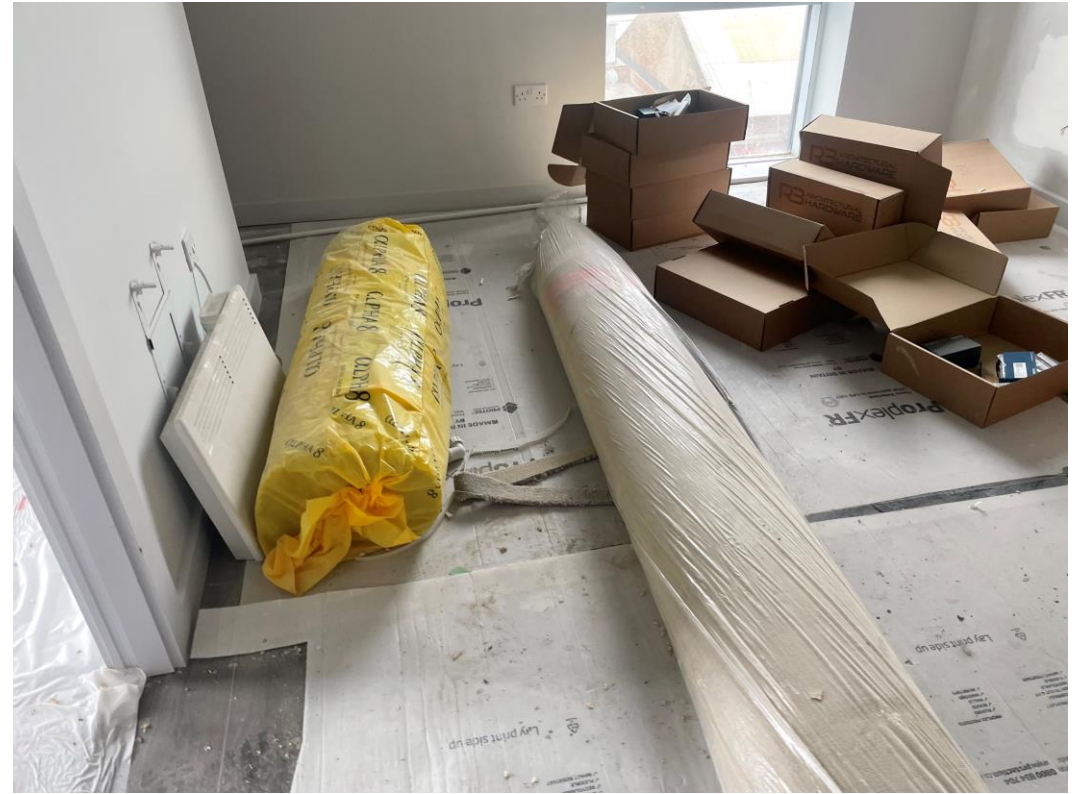
Carpets loaded for installation
