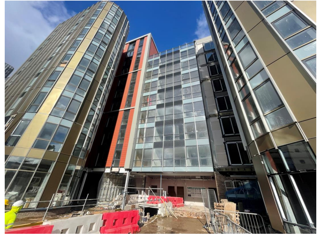
External cladding remedial works
