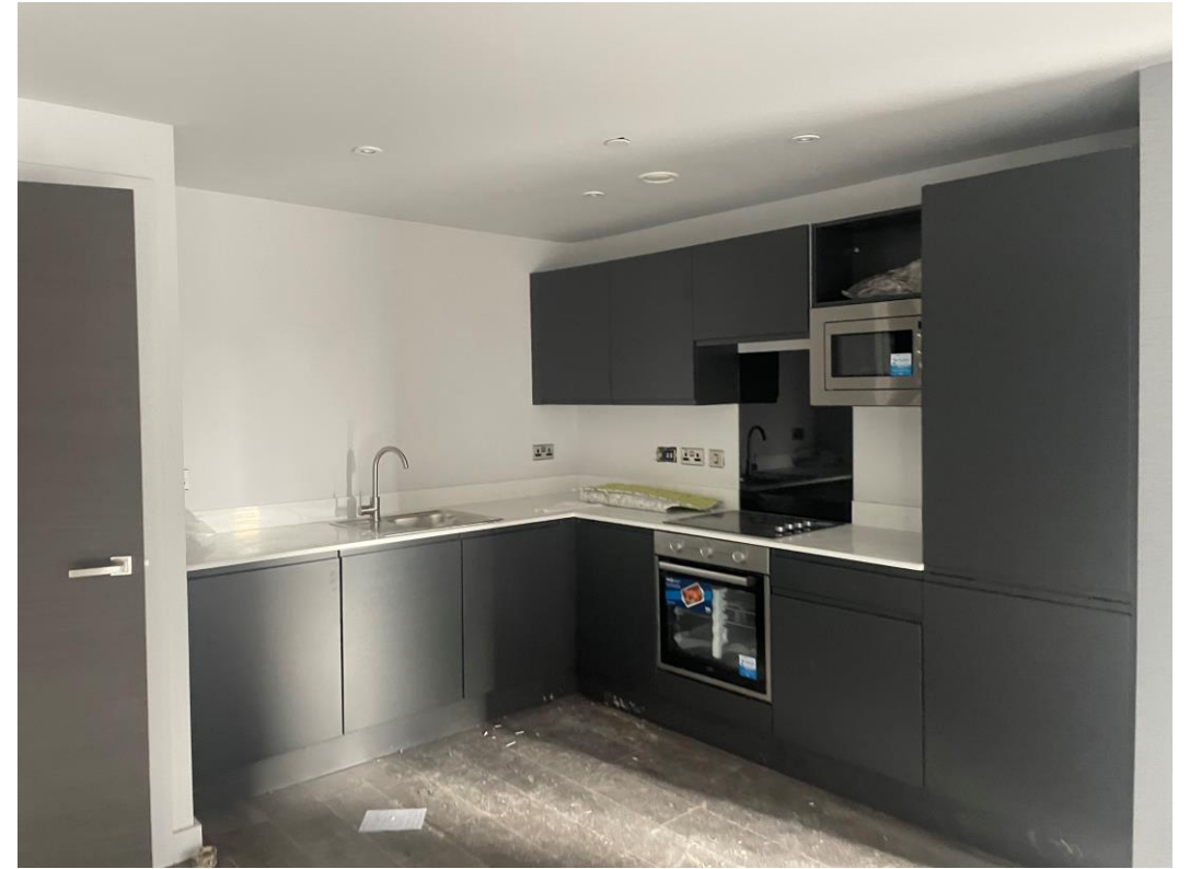
Block A – Kitchens installed
