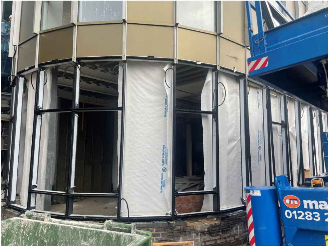
Curtain wall installation
