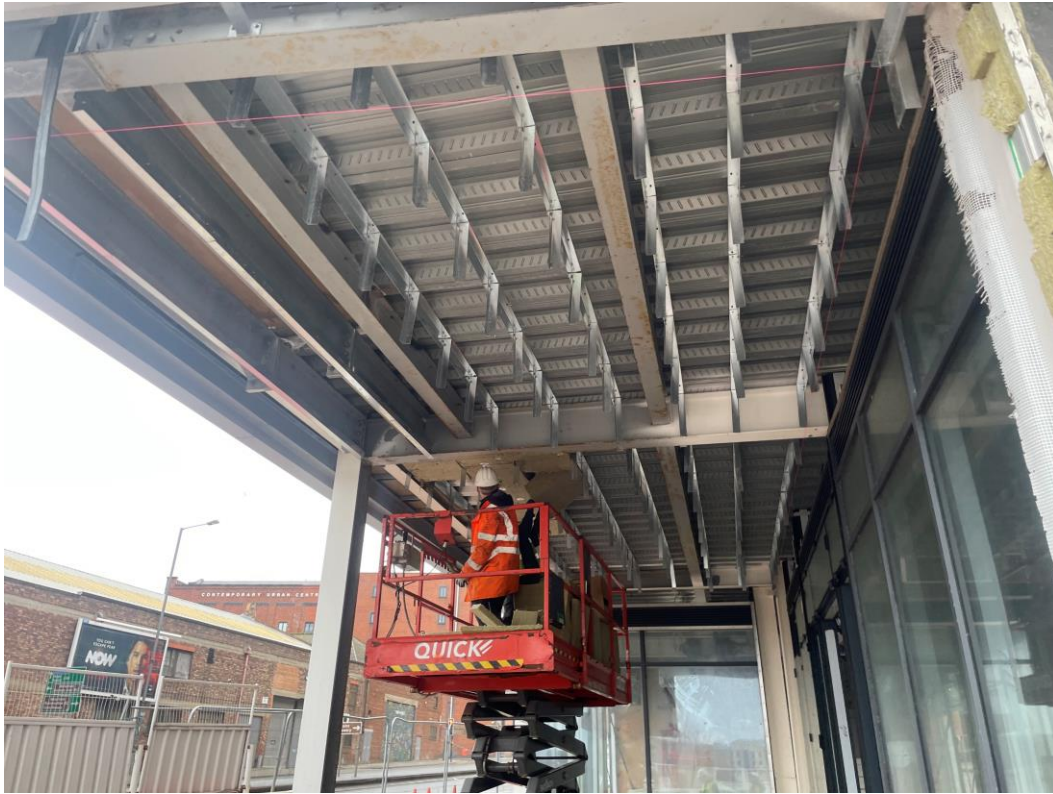
Soffit cladding rail installed
