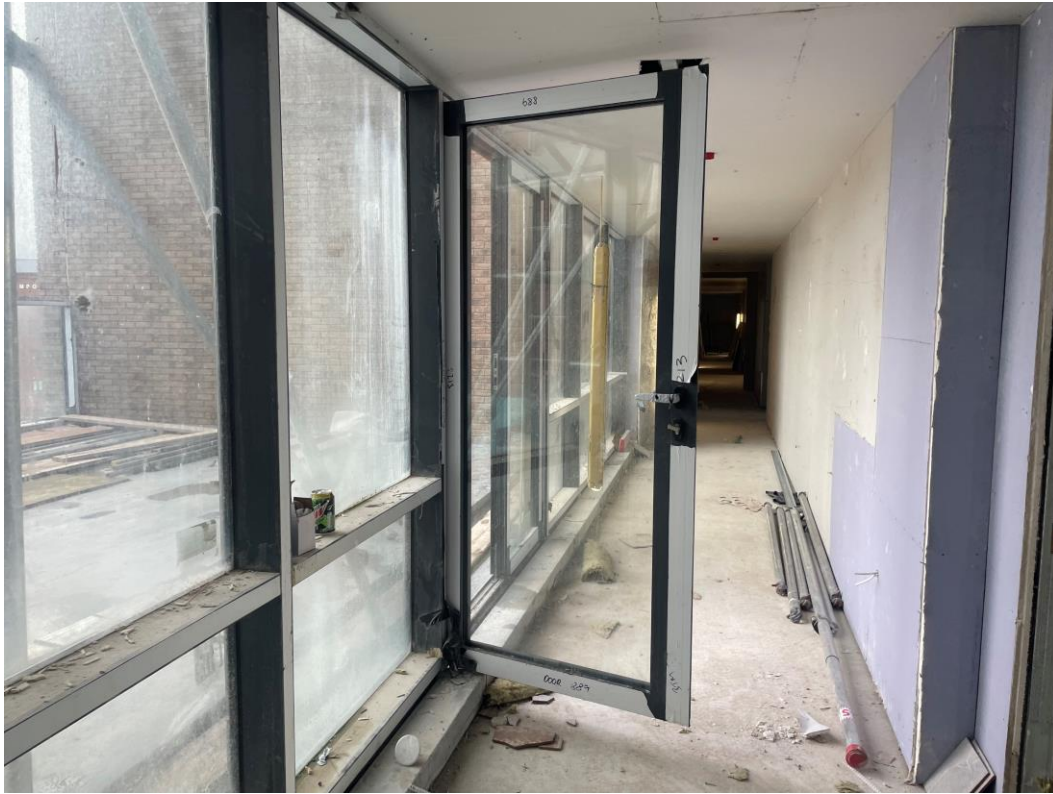
Doors installed for terrace link roof access
