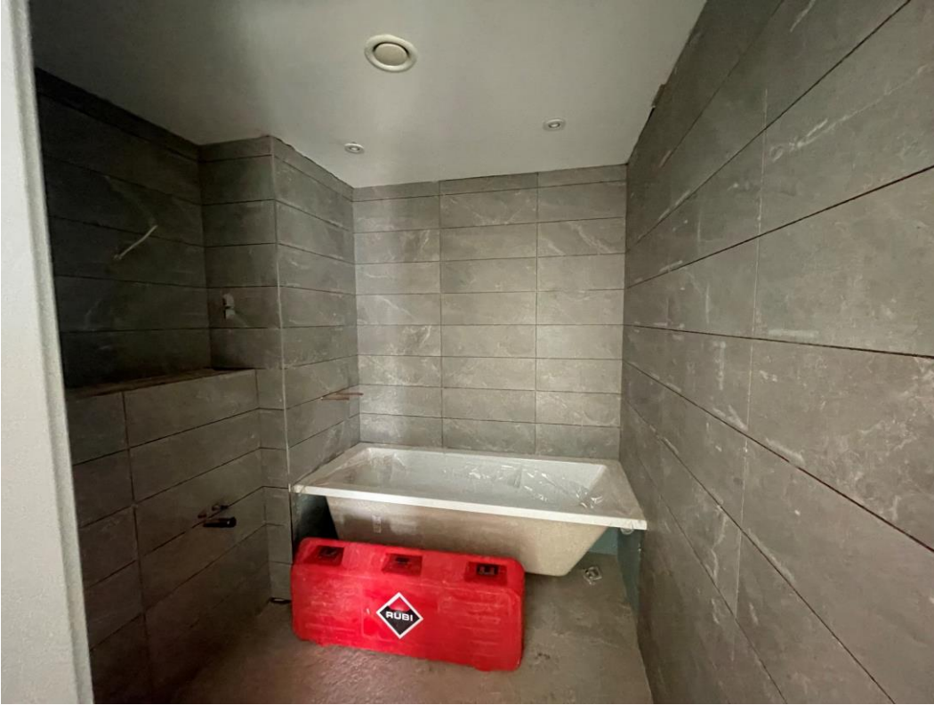
Installation of bathroom appliances ongoing
