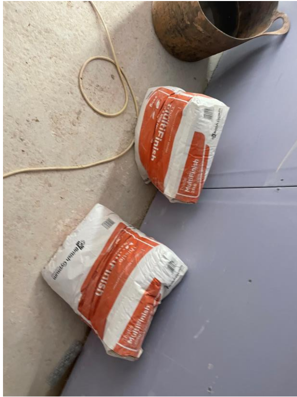
Plaster loaded for application
