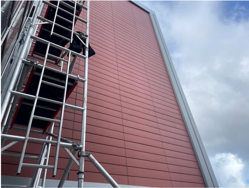
External cladding remedial works
