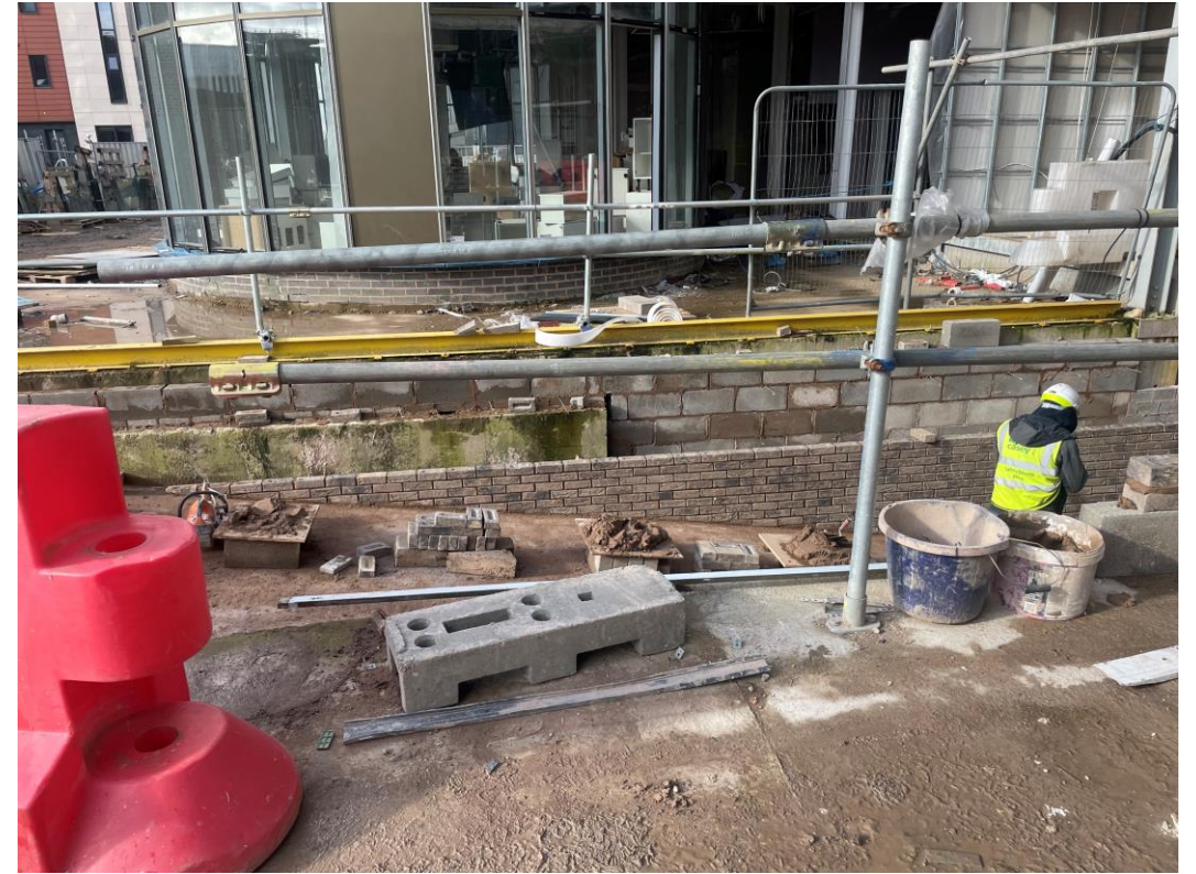
Brickwork installation to basement ramp
