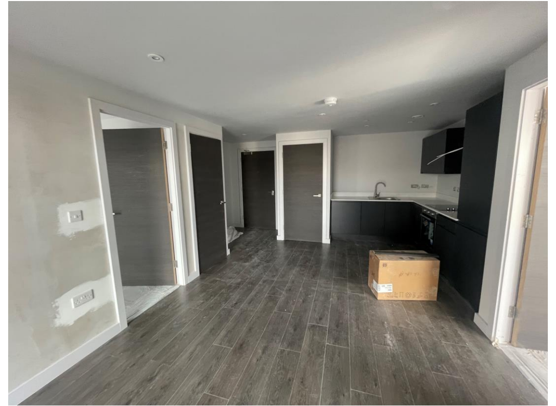
Block A - apartment doors & ironmongery installed
