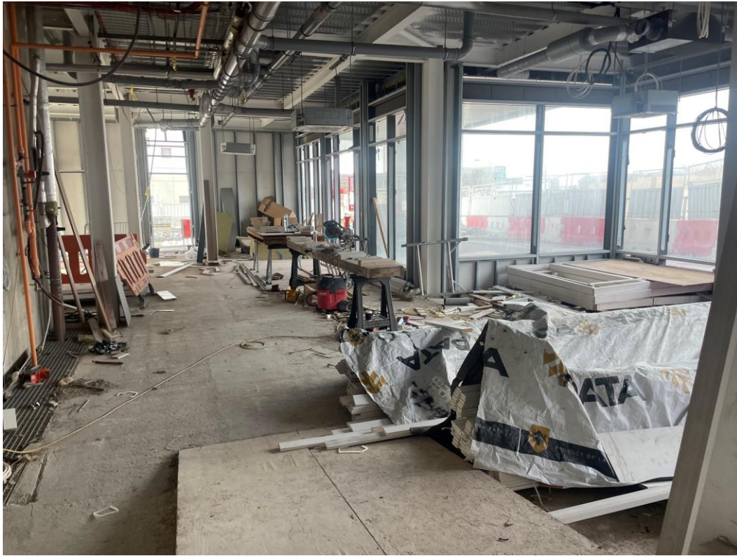
Ground Floor site activity
