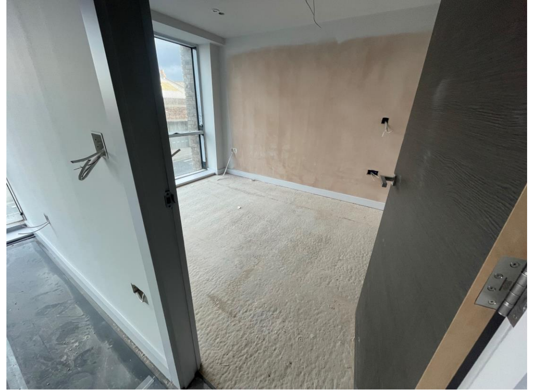
Apartment doors & ironmongery installed
