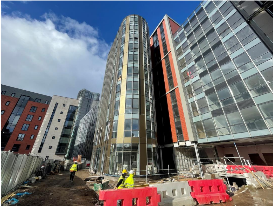
External cladding remedial works
