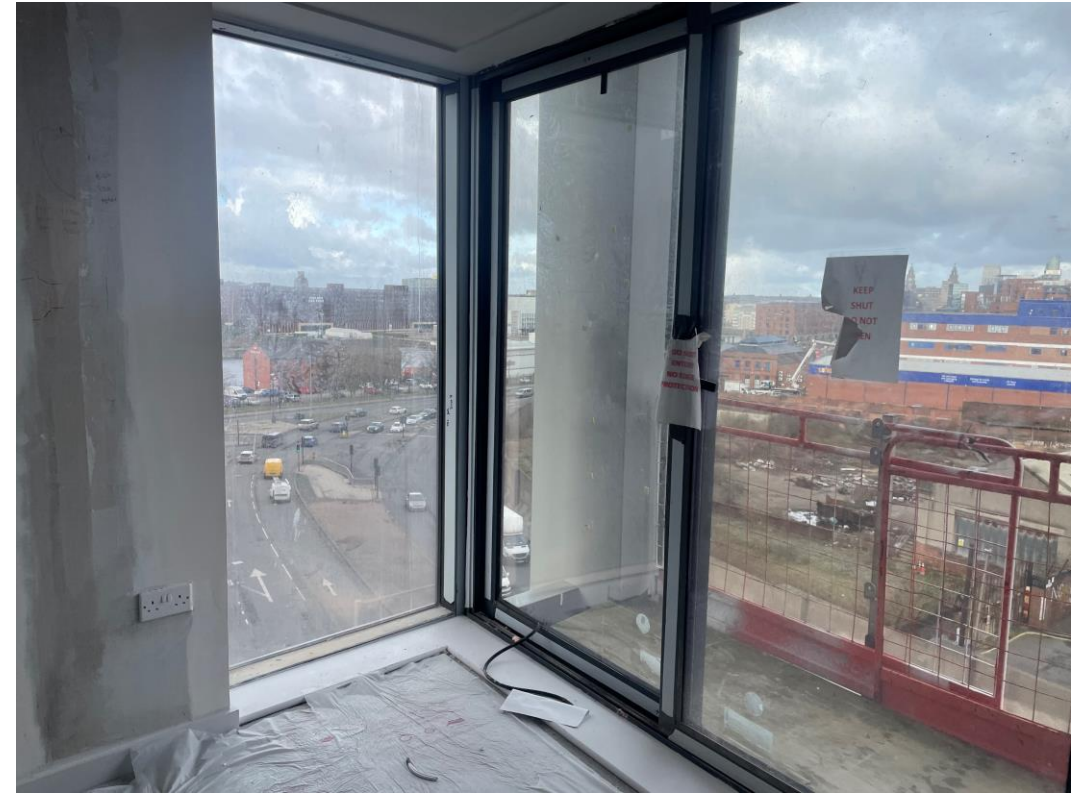
Apartment decoration ongoing
