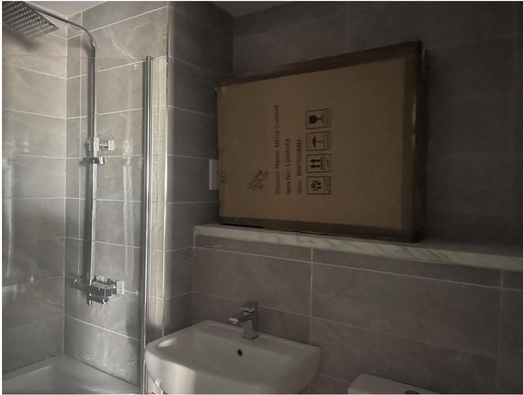
Bathroom mirrors installed
