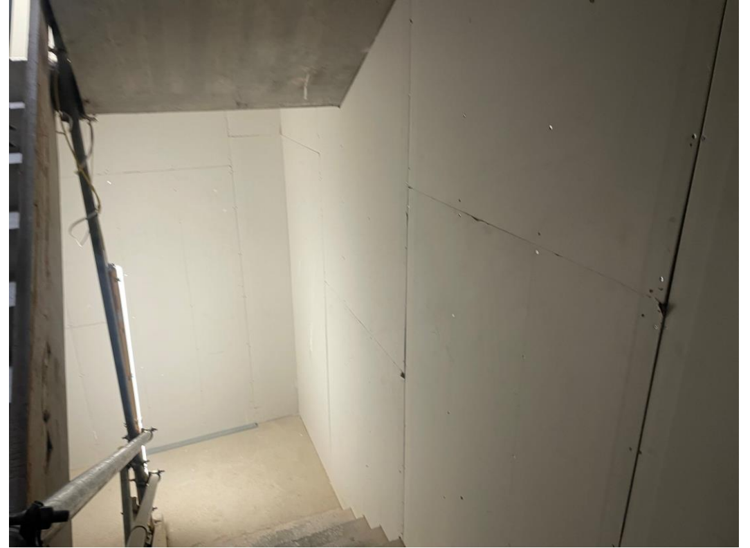
Stairwell wall boarding installed
