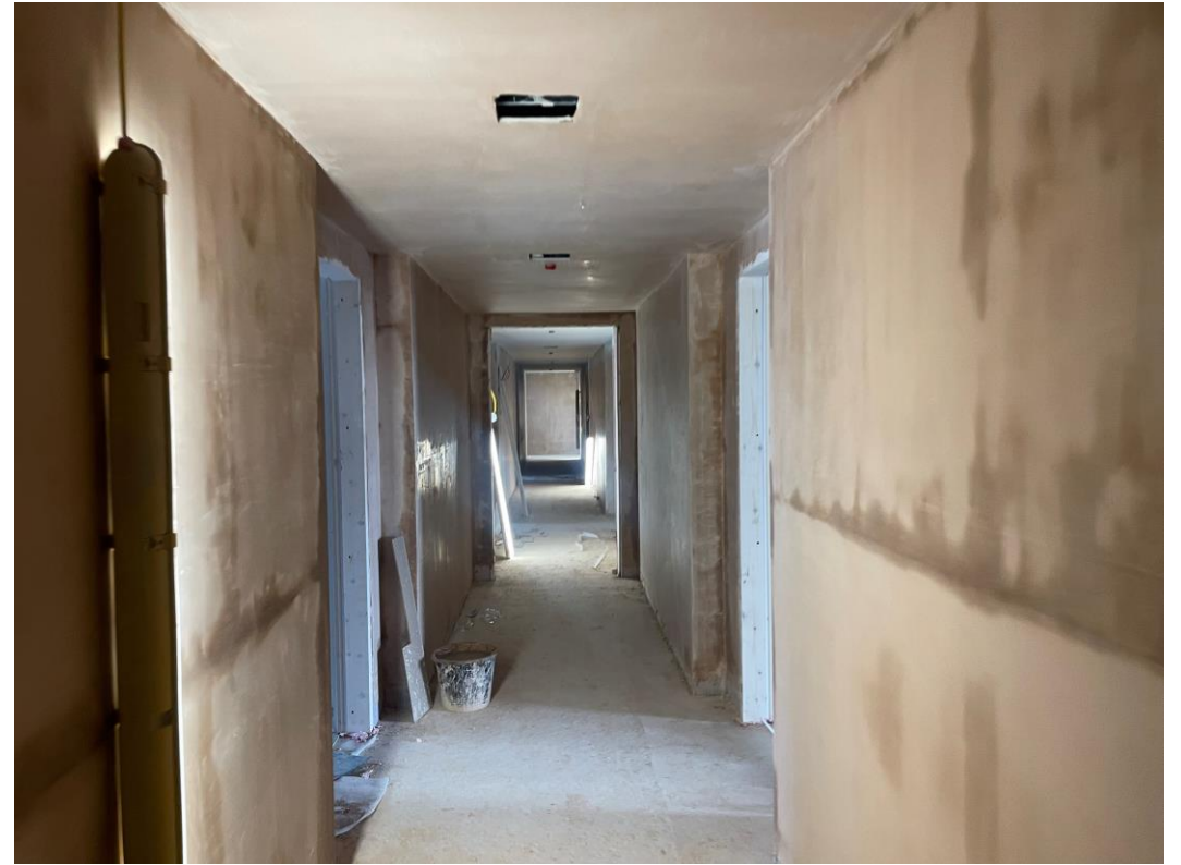
Walls skimmed to circulation areas
