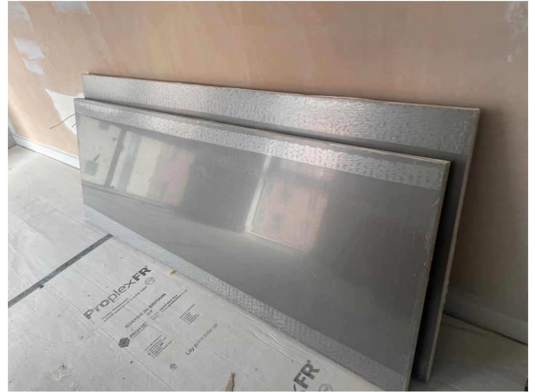
Doors loaded for installation
