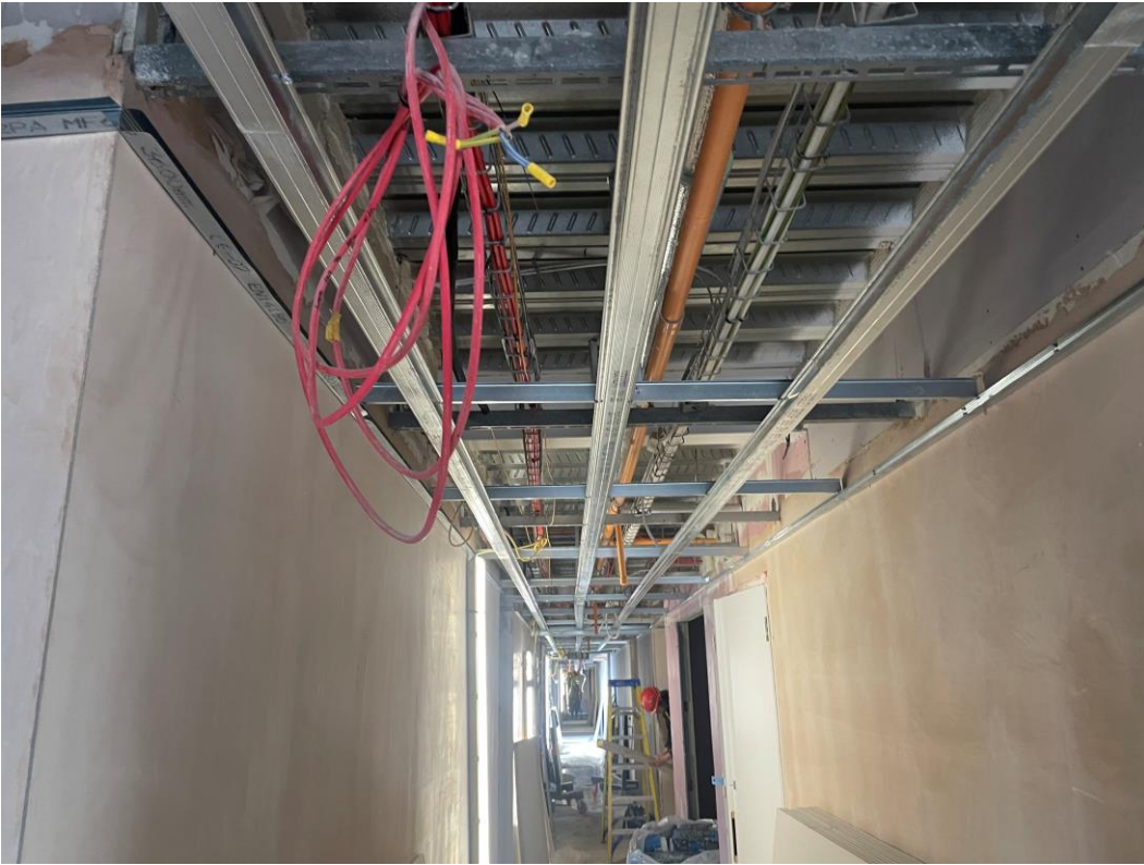
Ceiling grid installed
