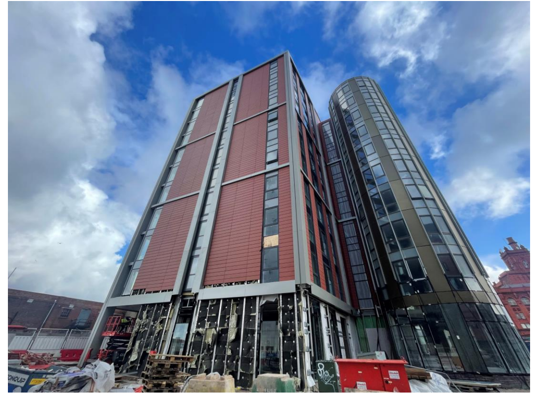
Caryl Street site view
