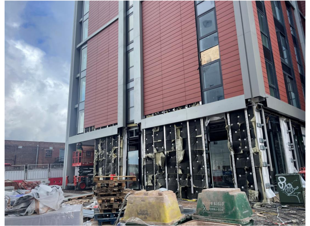
External cladding remedial works
