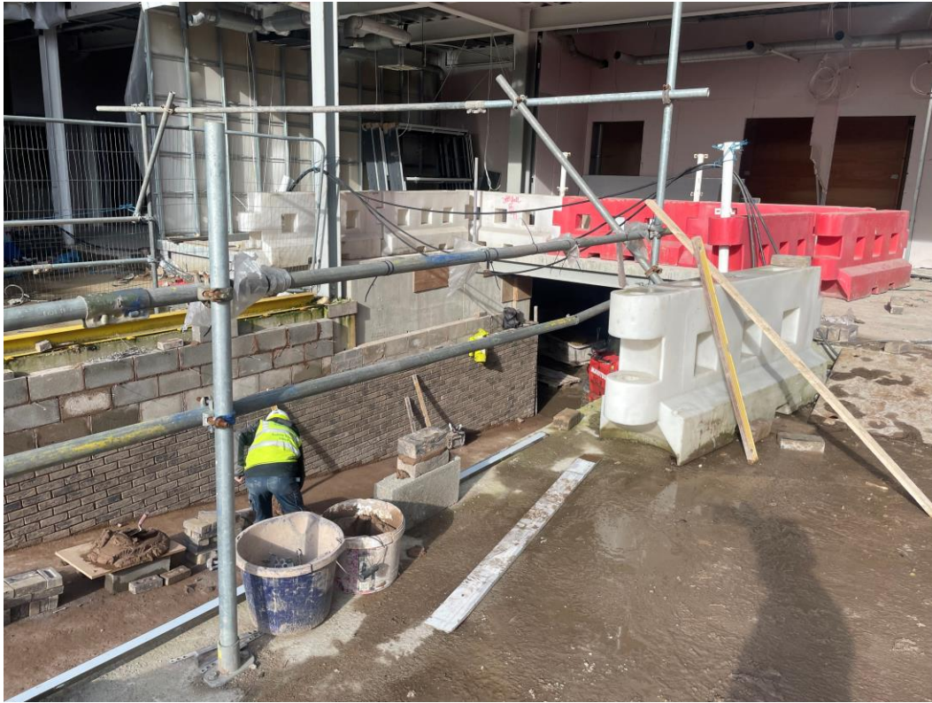
Brickwork installation to basement ramp
