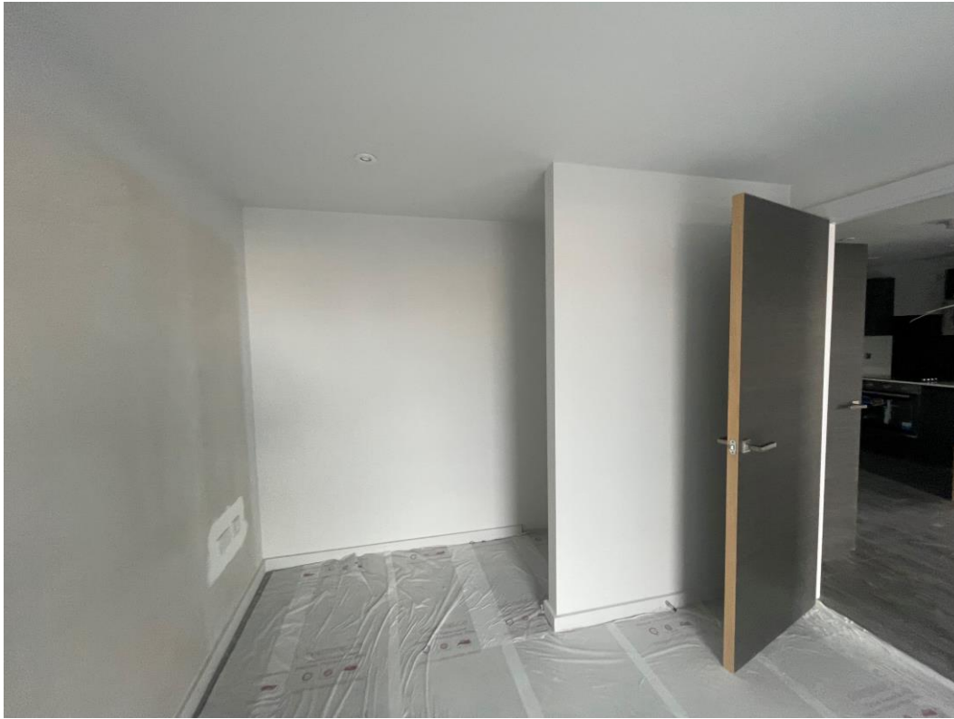
Apartment decoration ongoing
