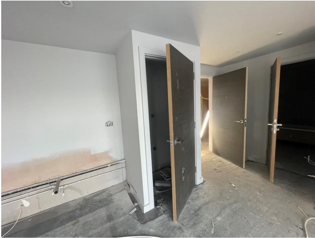
Apartment doors & ironmongery installed
