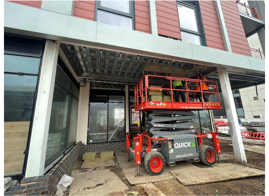
External cladding installation
