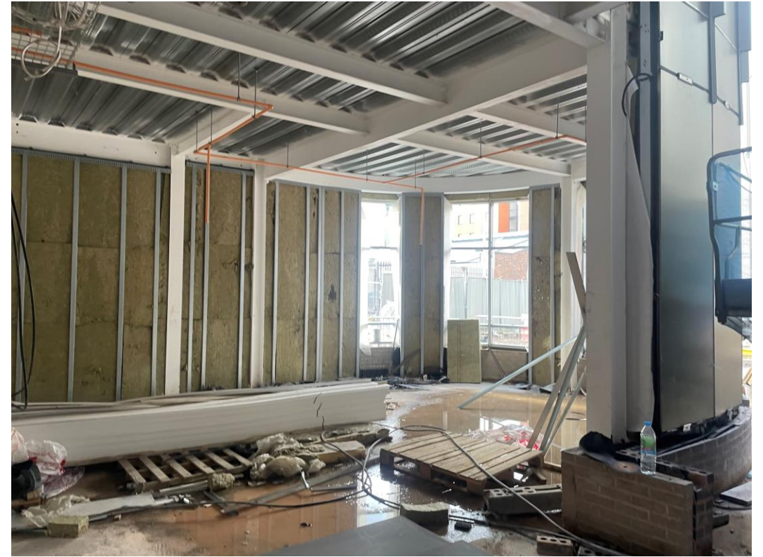
Ground Floor site activity
