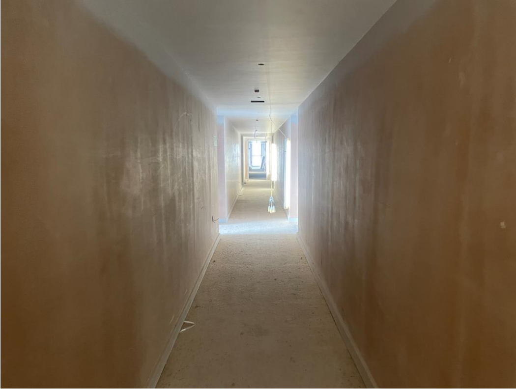
Walls & ceilings skimmed to circulation areas
