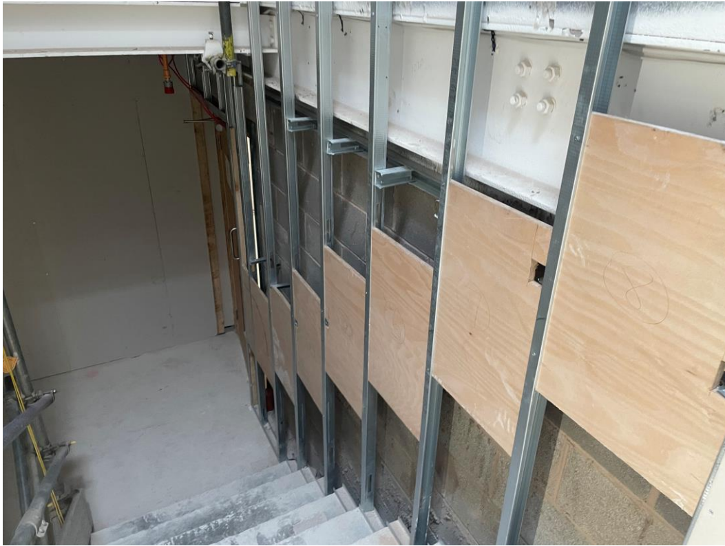
Partition & pattrass installed to stairwell
