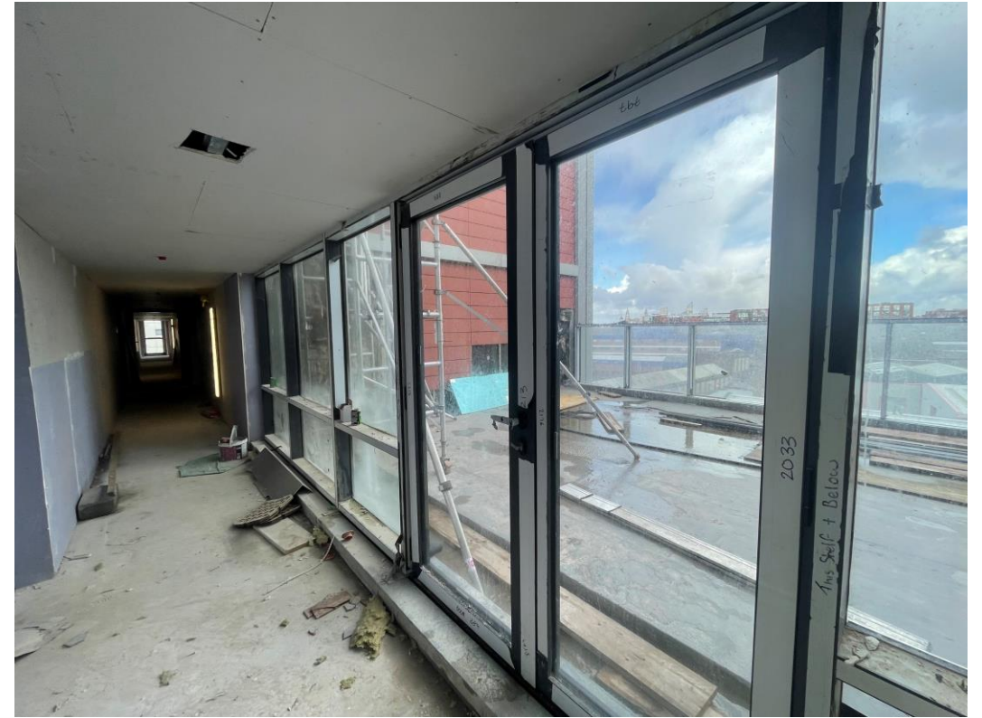
Doors installed for terrace link roof access
