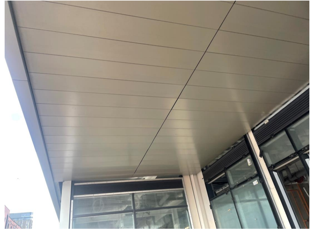
Soffit rain screen cladding installed
