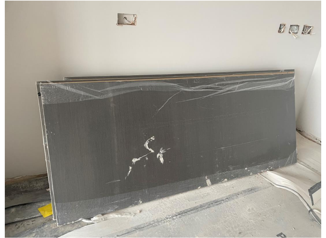
Doors loaded for installation
