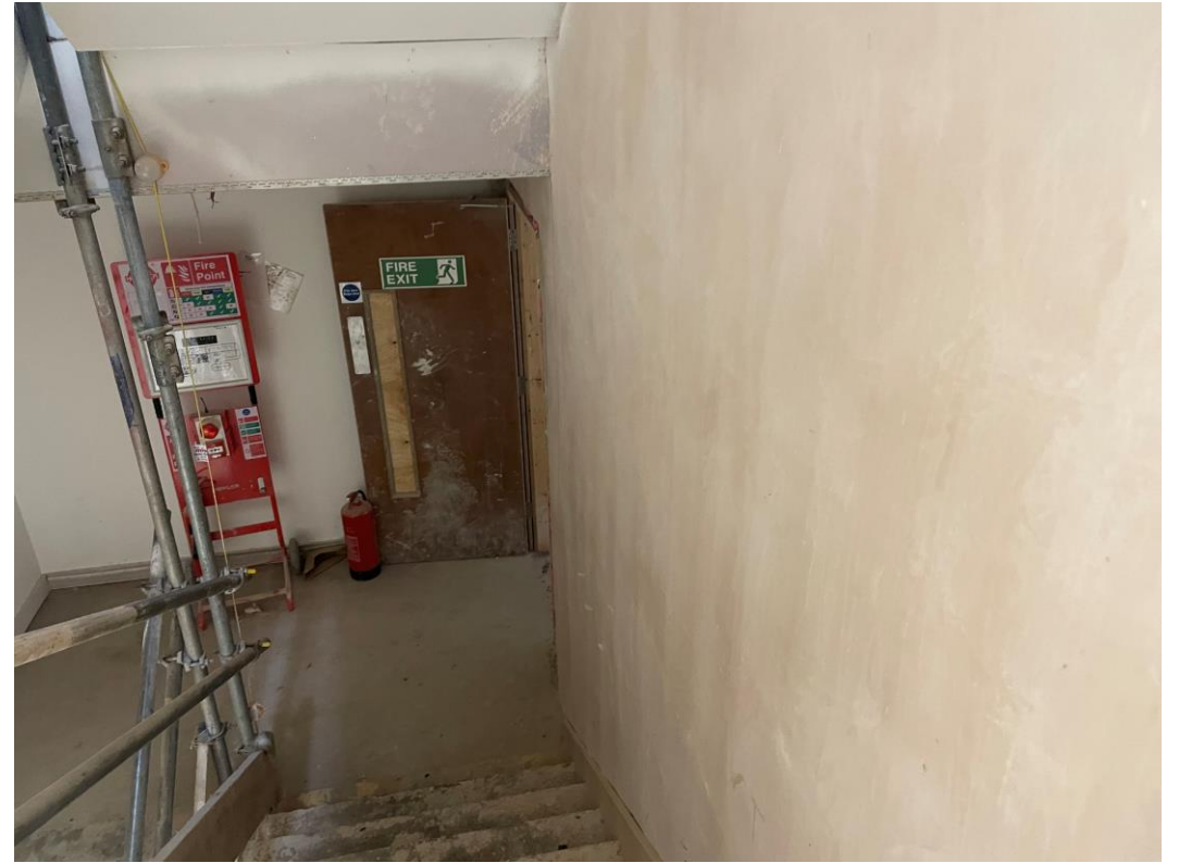
Walls plastered to stairwell
