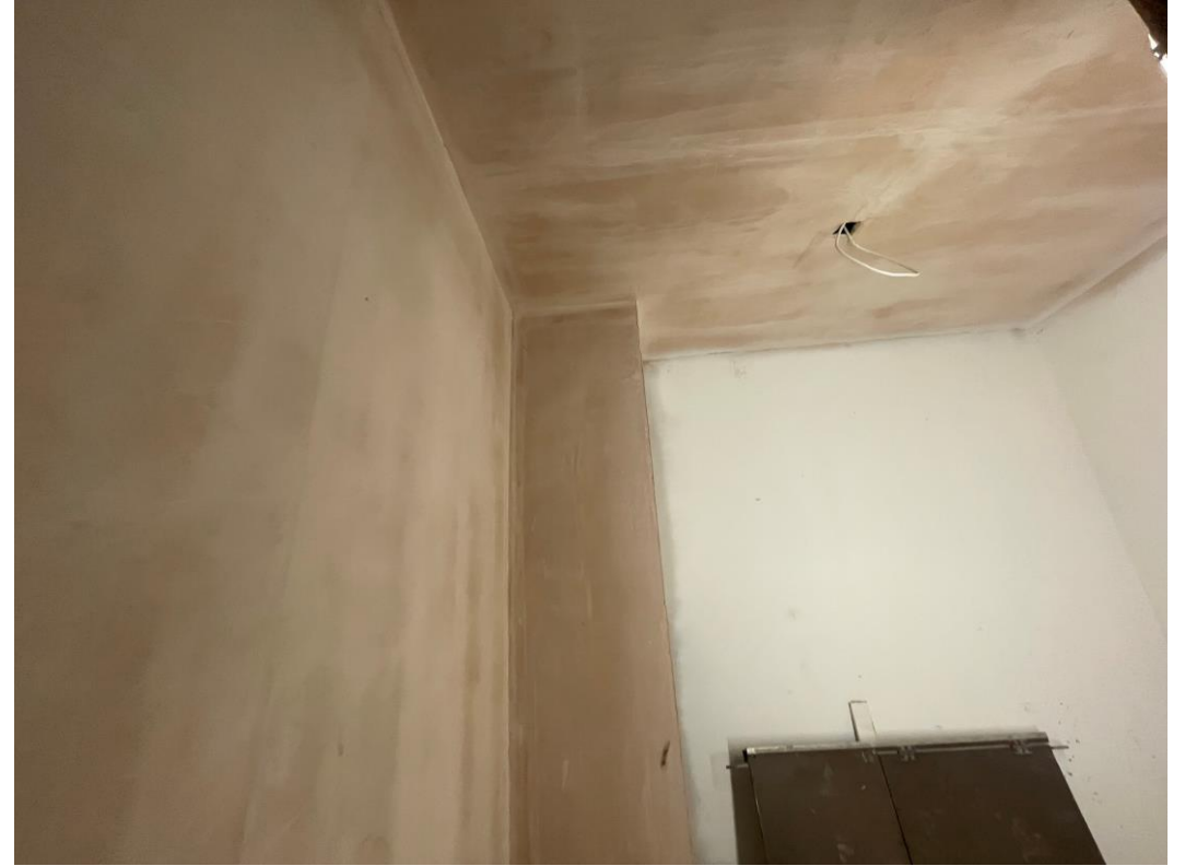
Walls & ceilings plastered to stairwell
