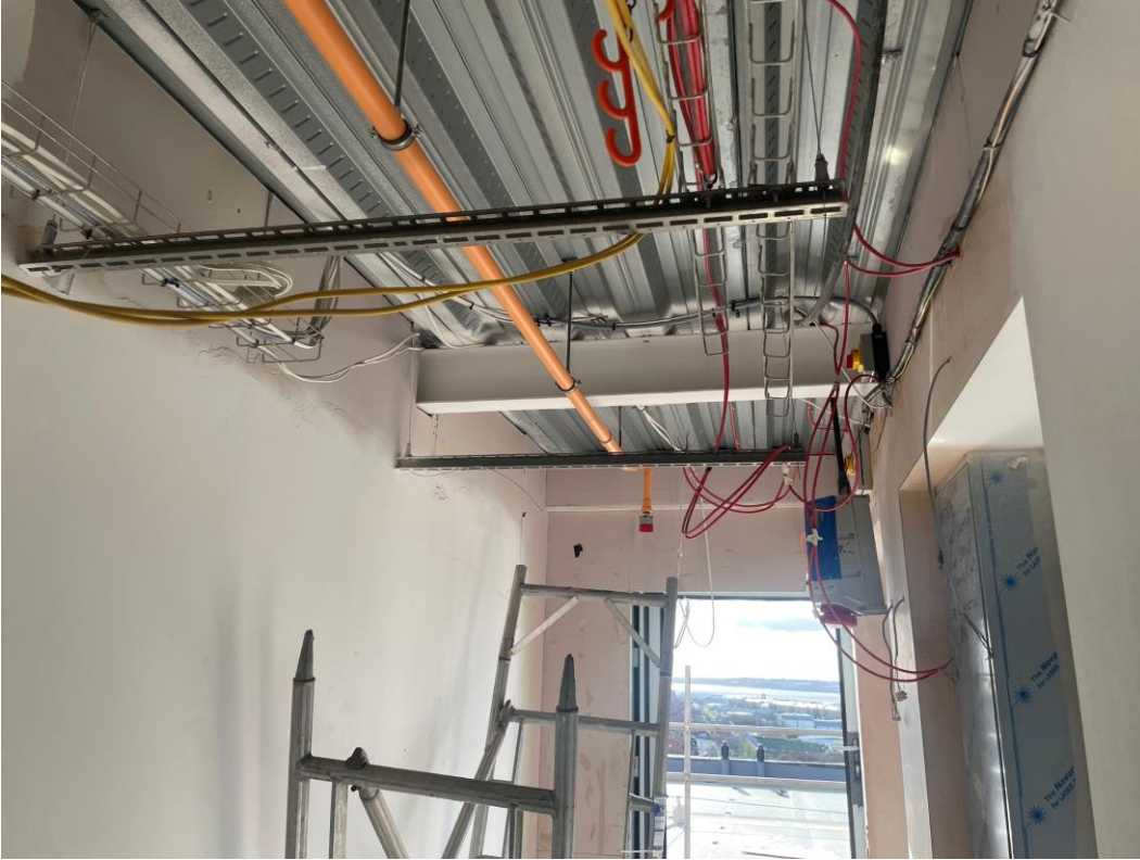
Sprinkler system installation
