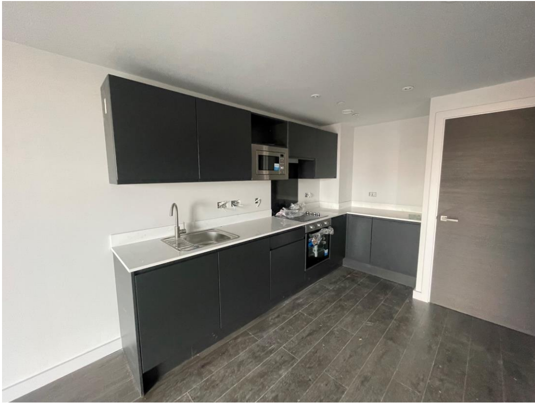
Block A – Kitchens installed
