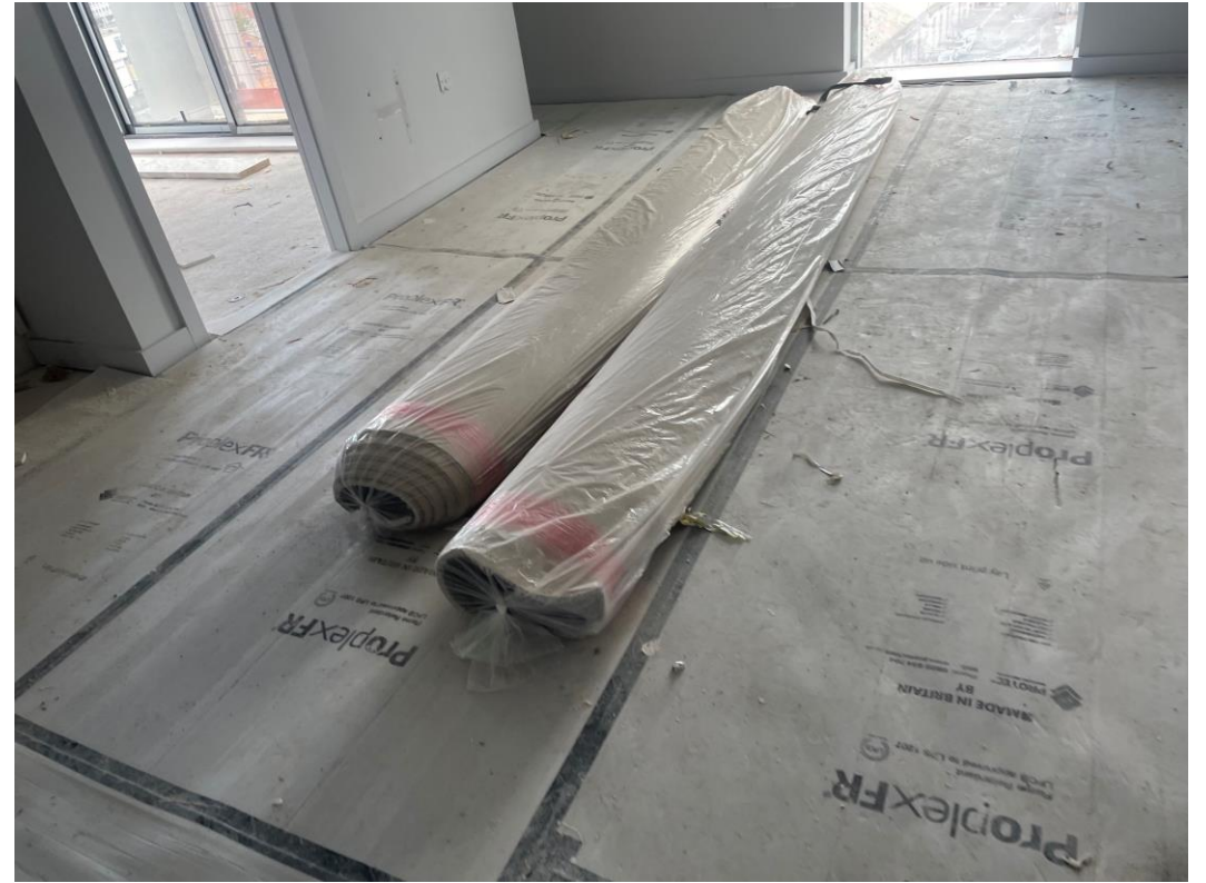
Carpets loaded for installation
