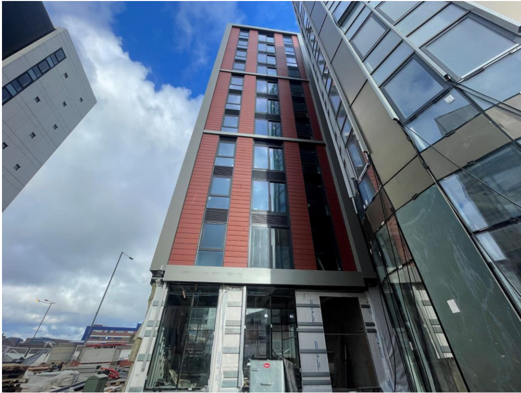
External cladding remedial works
