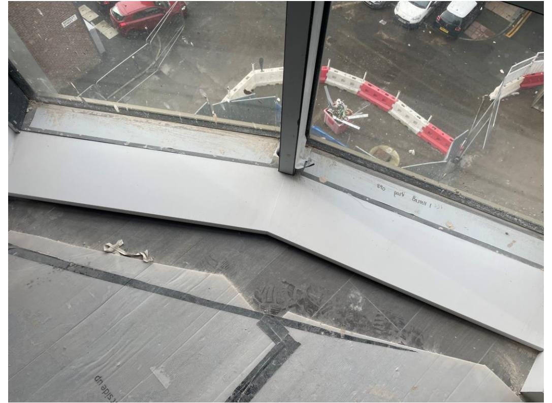
Window boards installed
