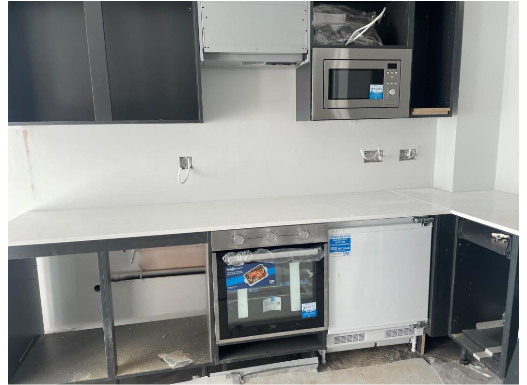
Kitchen unit installation
