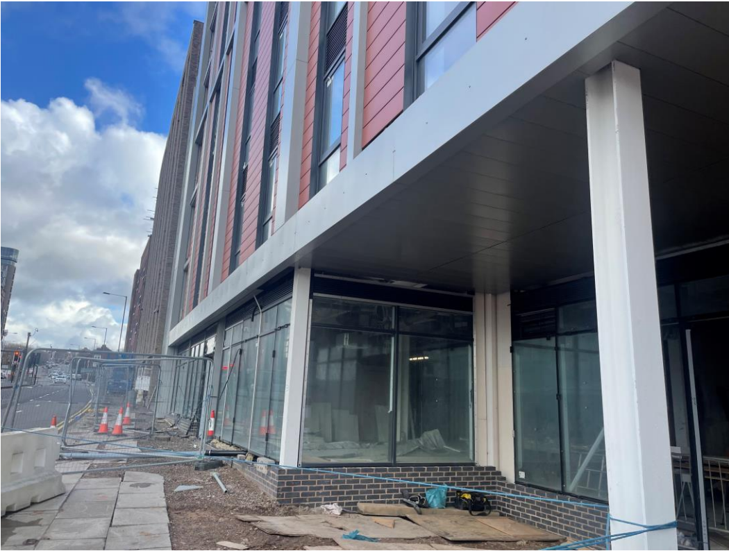
External cladding remedial works
