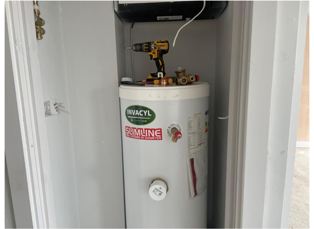
Installation of water cylinder ongoing
