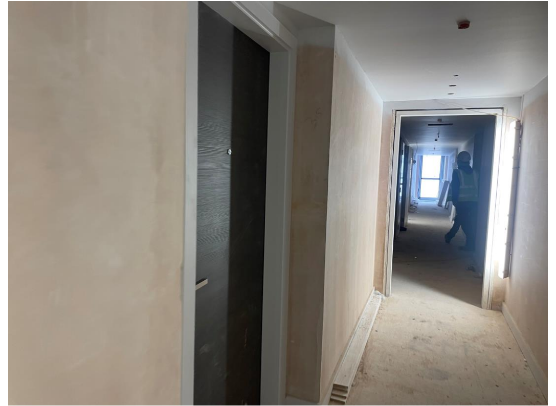
Apartment doors installed
