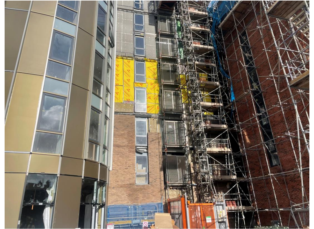
Brindley Street elevation insulation & brickwork ongoing
