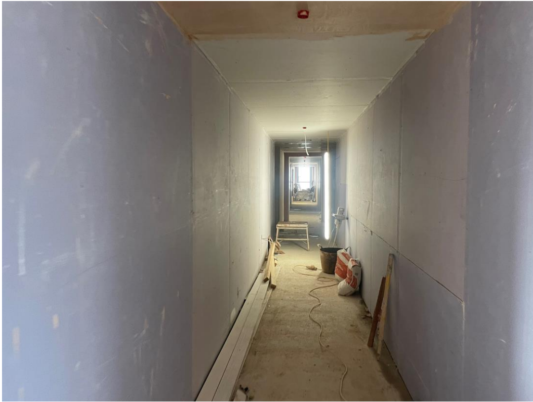
Walls boarded to circulation areas
