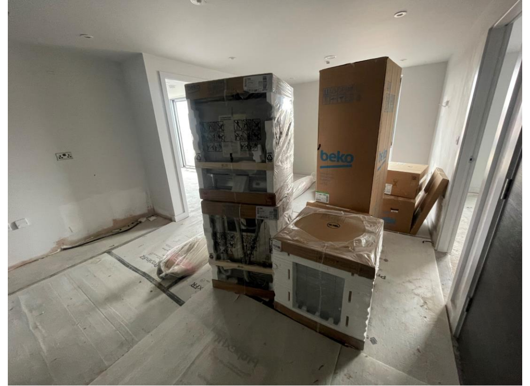
Appliances loaded for installation
