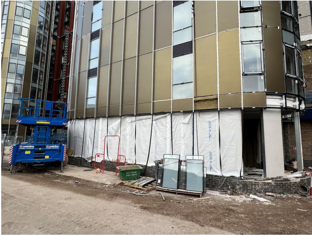
Curtain walling installation to ground level
