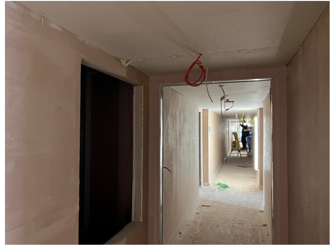
Block B – Walls skimmed to corridors
