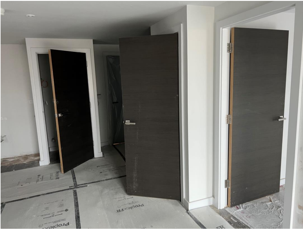
Apartment doors installed
