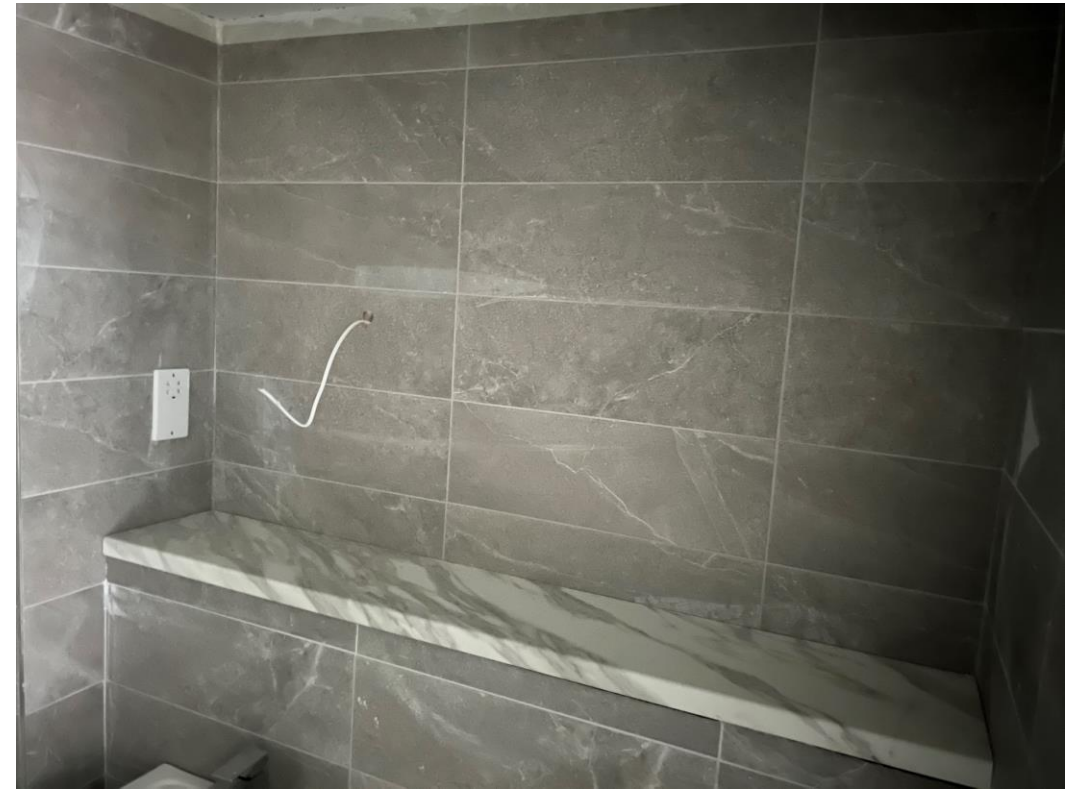
Bathroom vanity shelf installed
