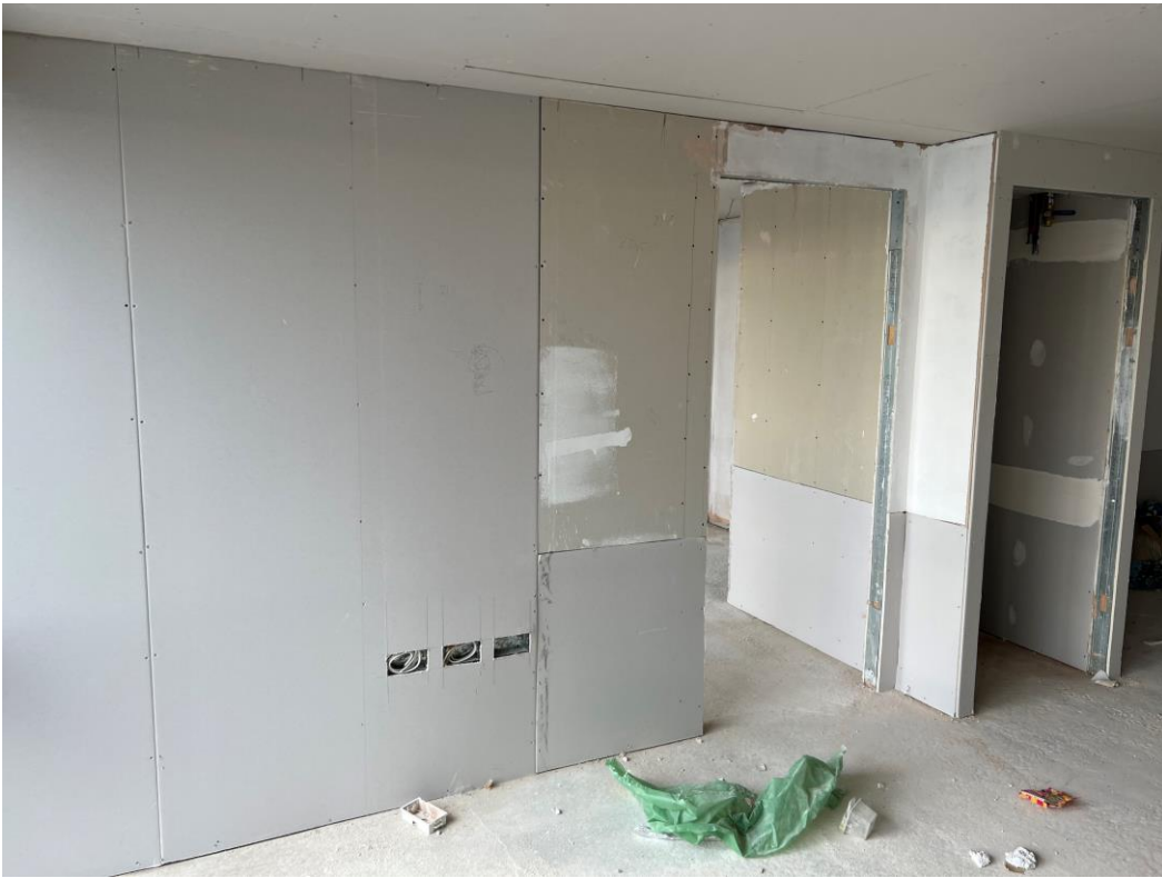
Plasterboard installed
