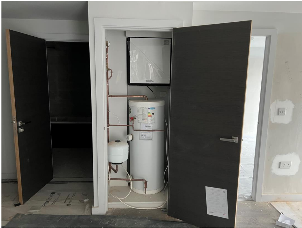
Water cylinder and ventilation unit installed
