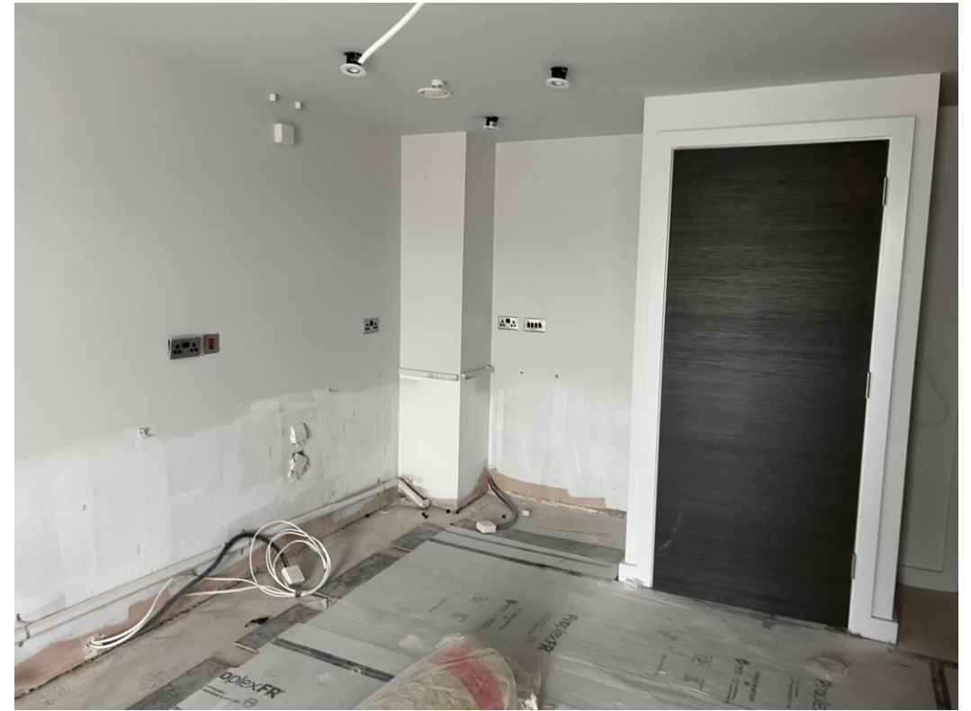
Apartment doors installed
