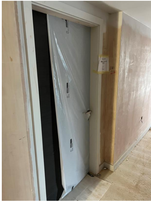
Apartment doors installed
