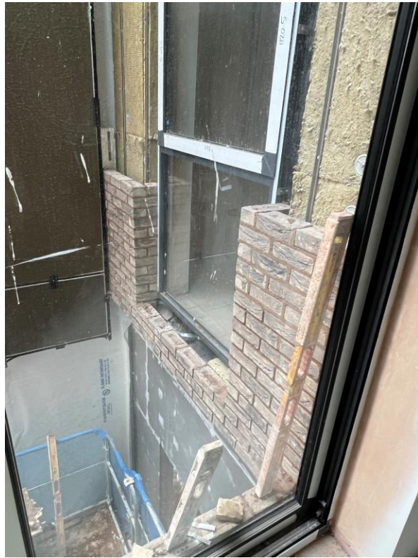
Brindley Steet Elevation – brickwork commenced
