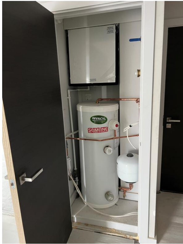
Water cylinder and ventilation unit installed
