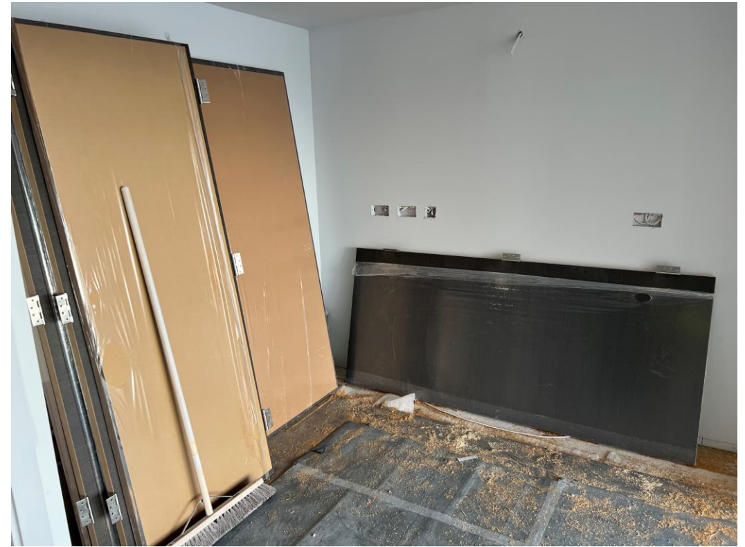
Doors loaded for installed
