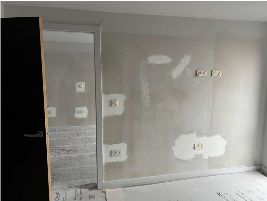
2 nd fix electrics completed to feature wall
