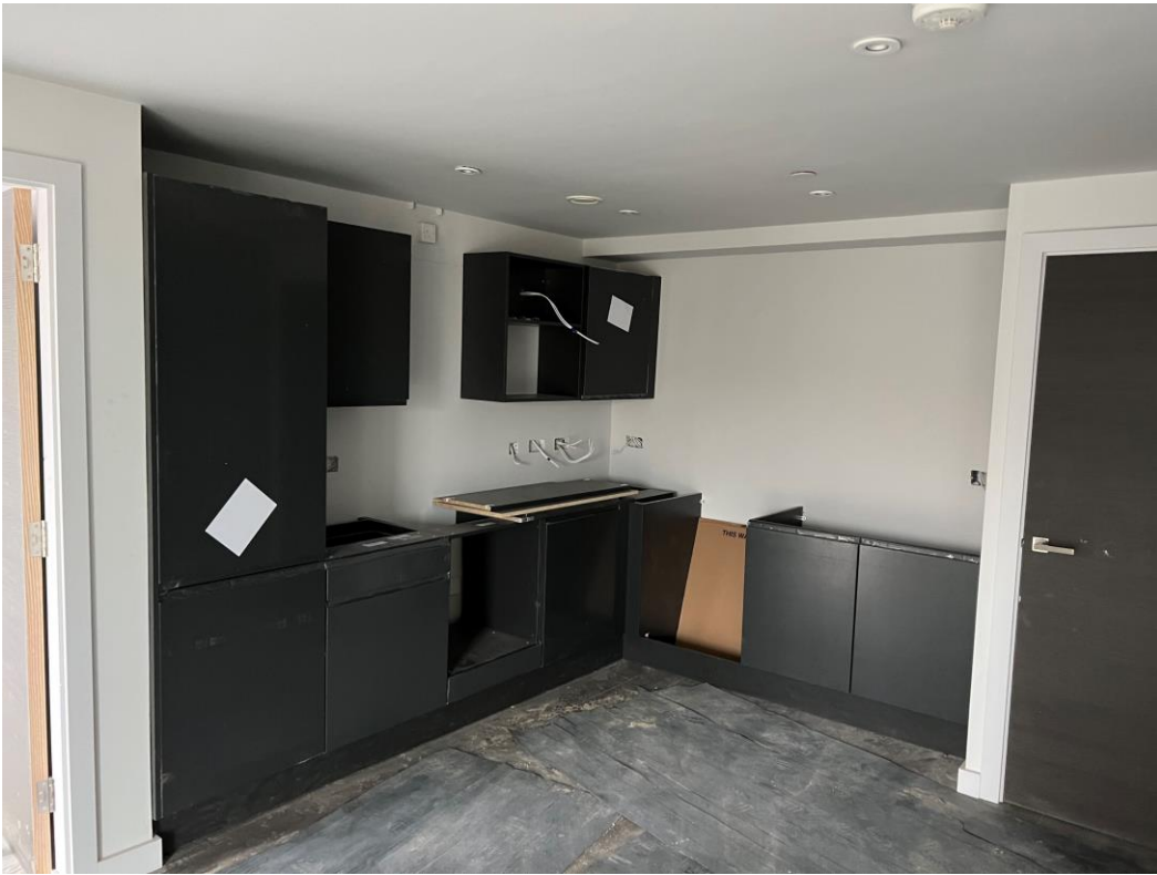
Block A – Kitchen units commenced
