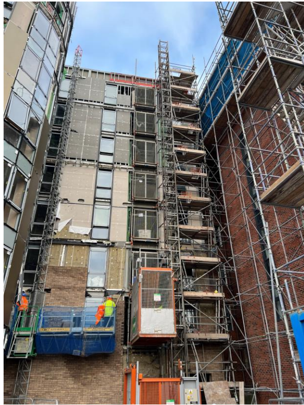
Brindley Steet Elevation brickwork commenced
