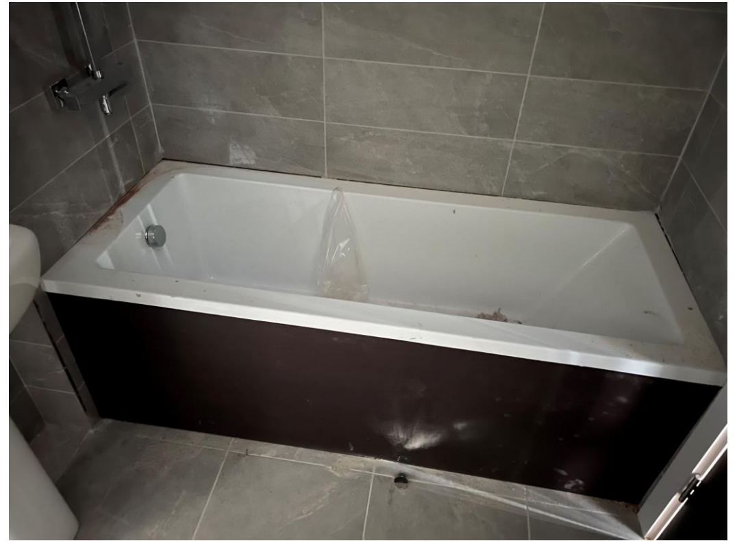
Bath & panel installed
