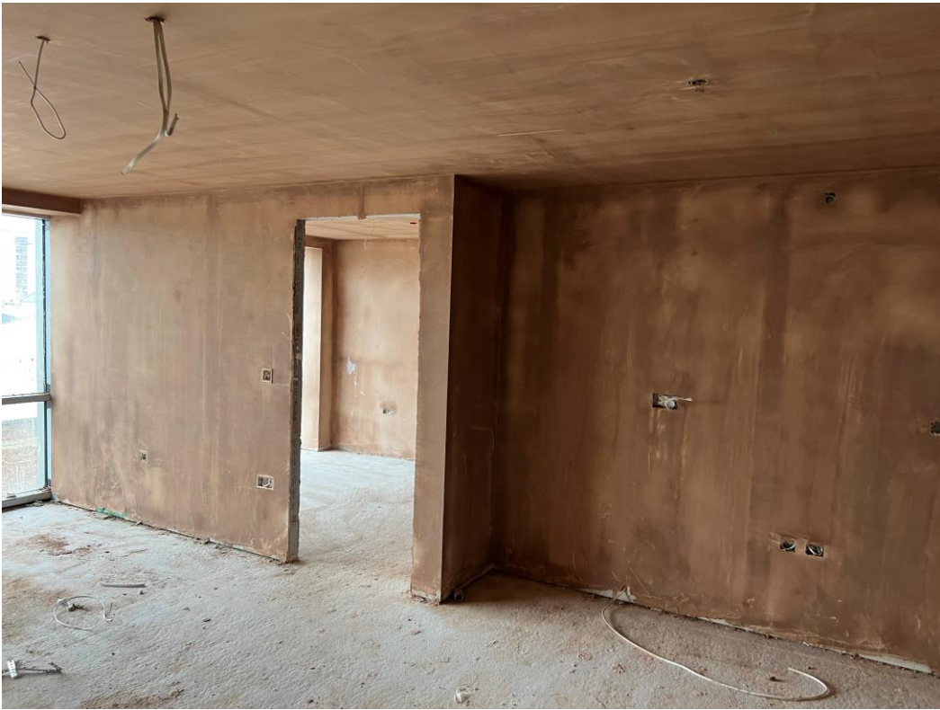
Apartment walls & ceilings plaster skimmed
