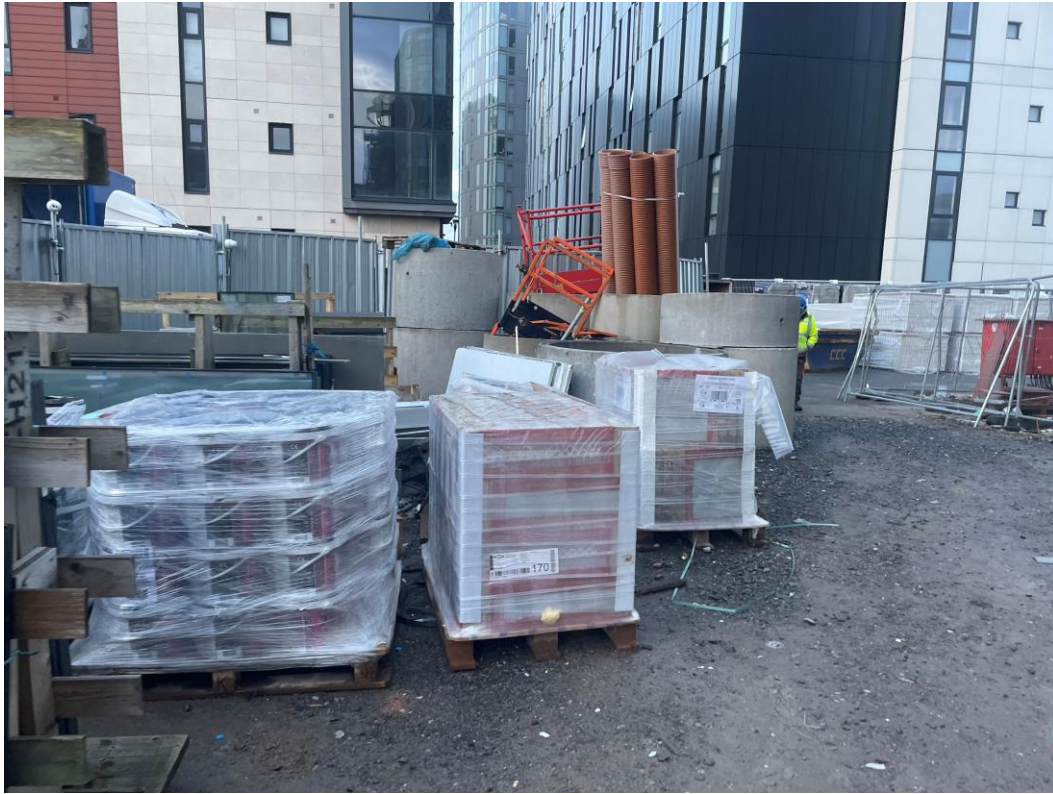
Tile & Tile Adhesive stored onsite
