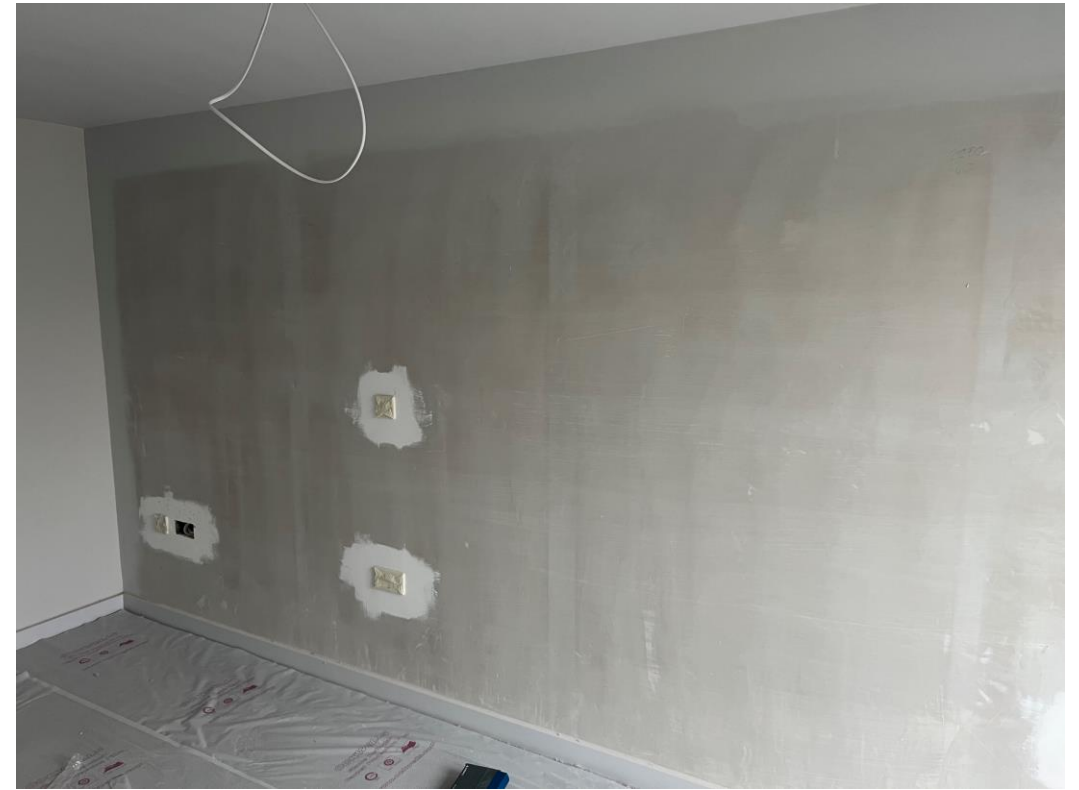
2 nd Fix electrics to feature wall
