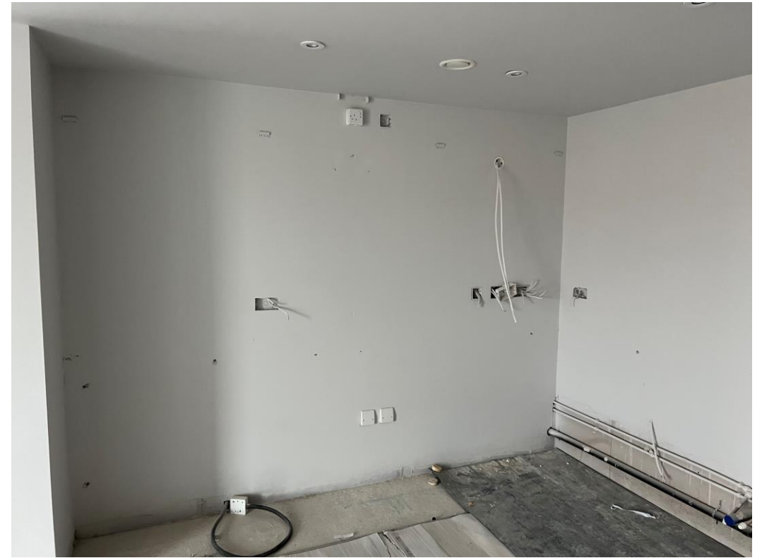
2 nd fix electrics to kitchen
