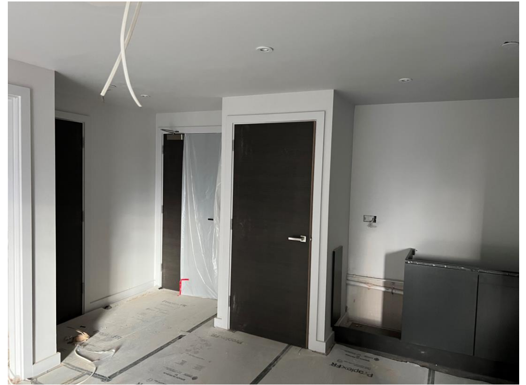
Apartment doors installed
