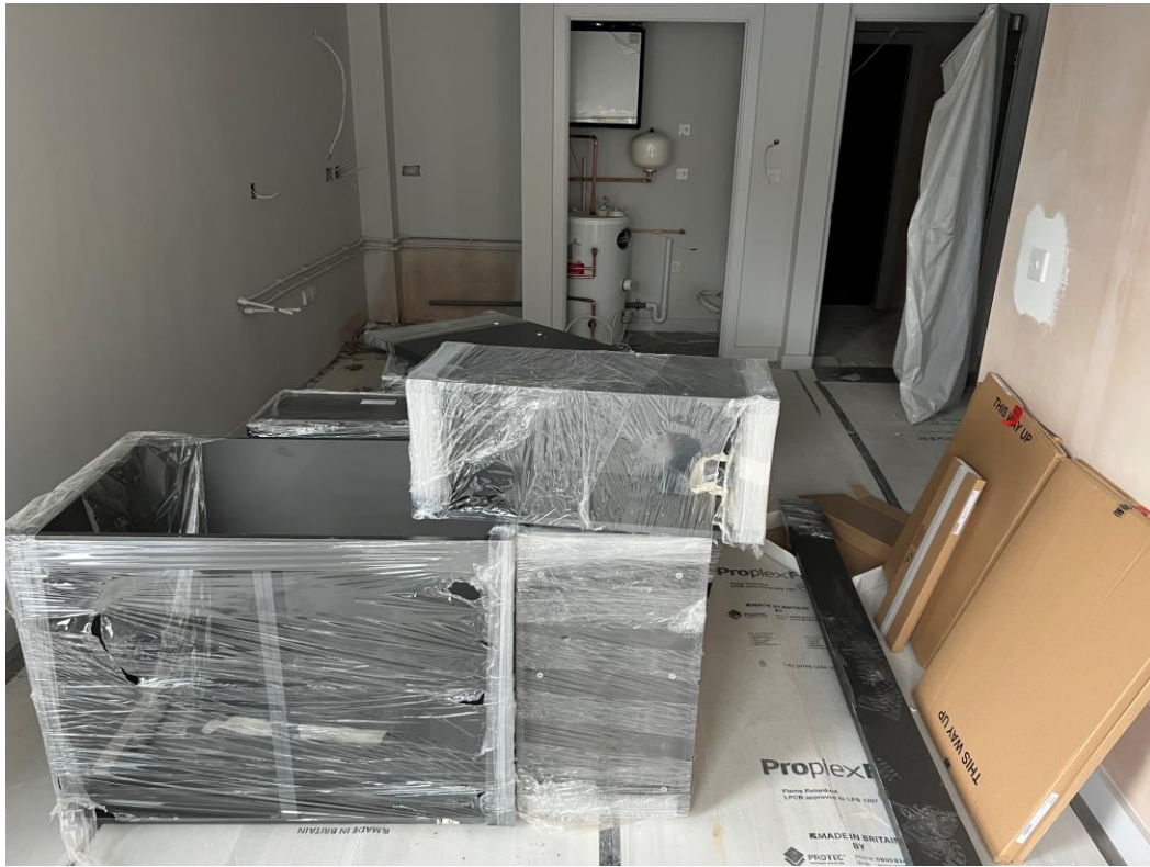
Kitchen units loaded for installation
