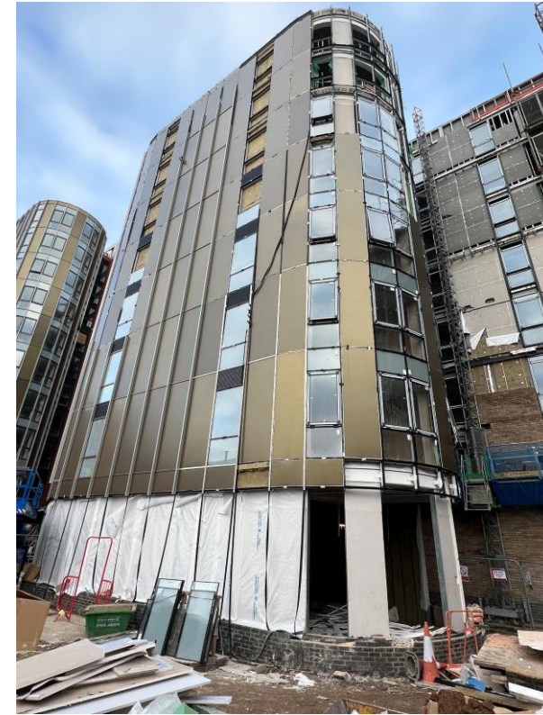
External cladding remedial works
