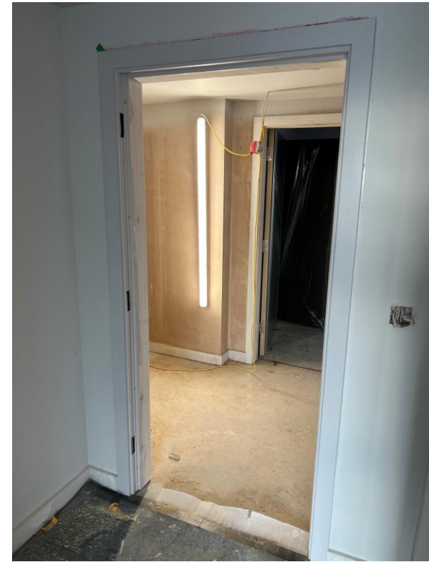
2 nd fix joinery installed
