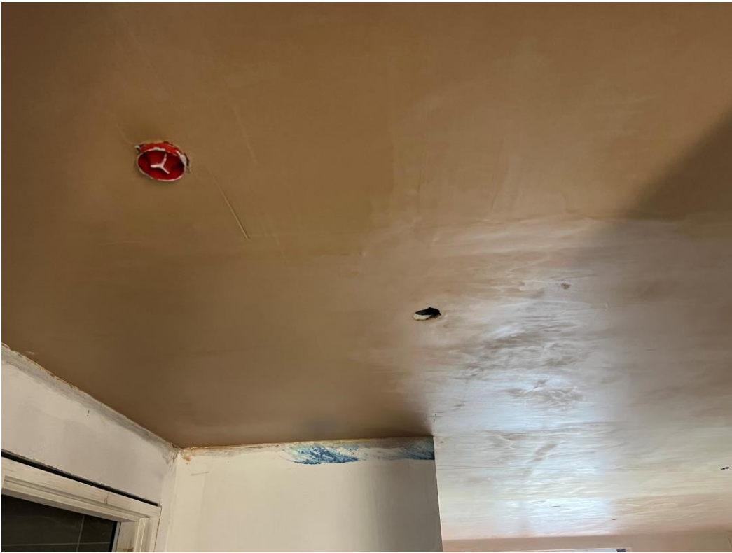
Ceilings plaster skimmed to apartments
