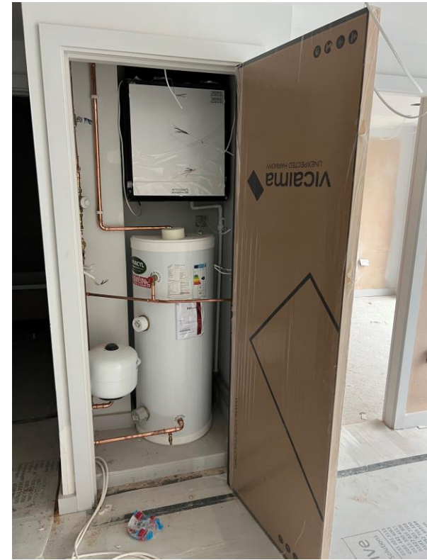
Water cylinder and ventilation unit installed
