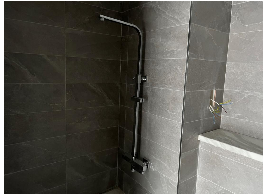
Shower bar installed
