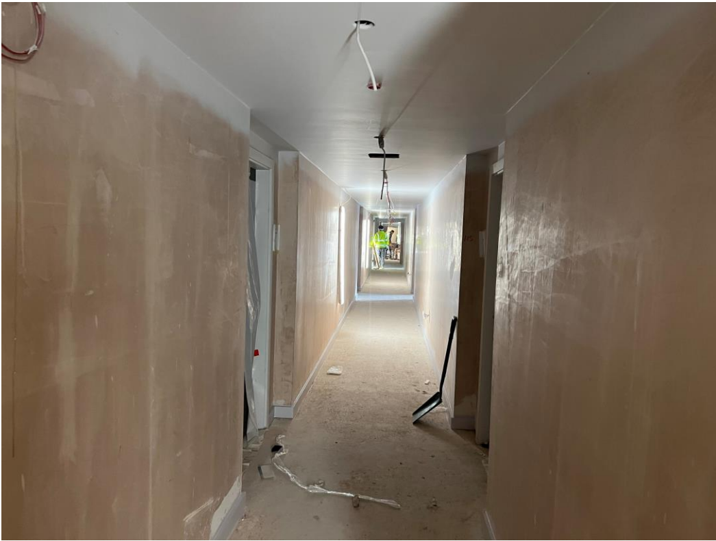
Block B – Ceilings skimmed to corridors
