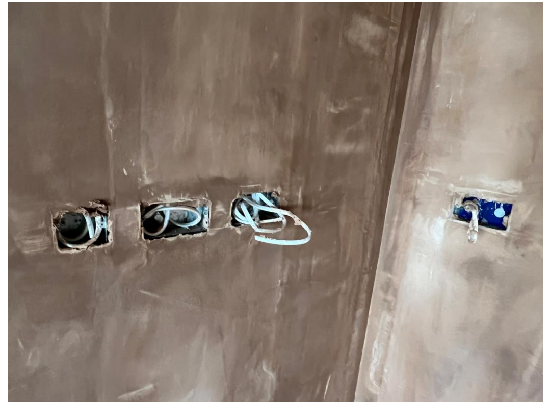
Walls plaster skimmed to apartments
