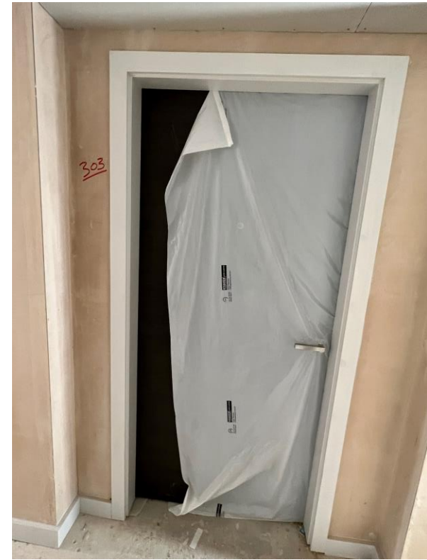
Apartment doors installed
