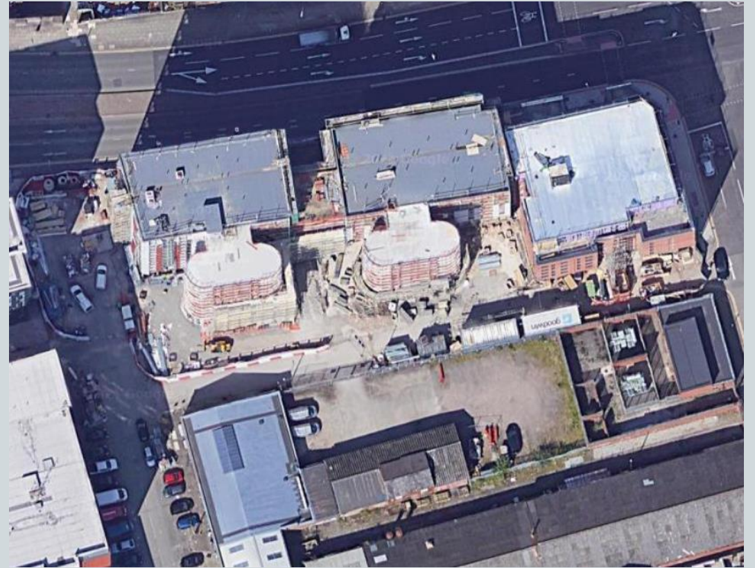
Aerial view of The Summit site location
