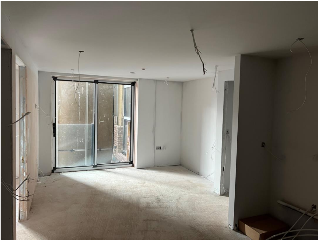
Decoration to apartment ceilings
