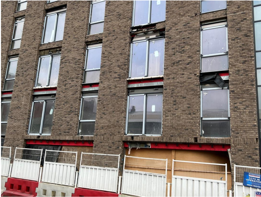
Brick remedial works to Parliament Street Elevation
