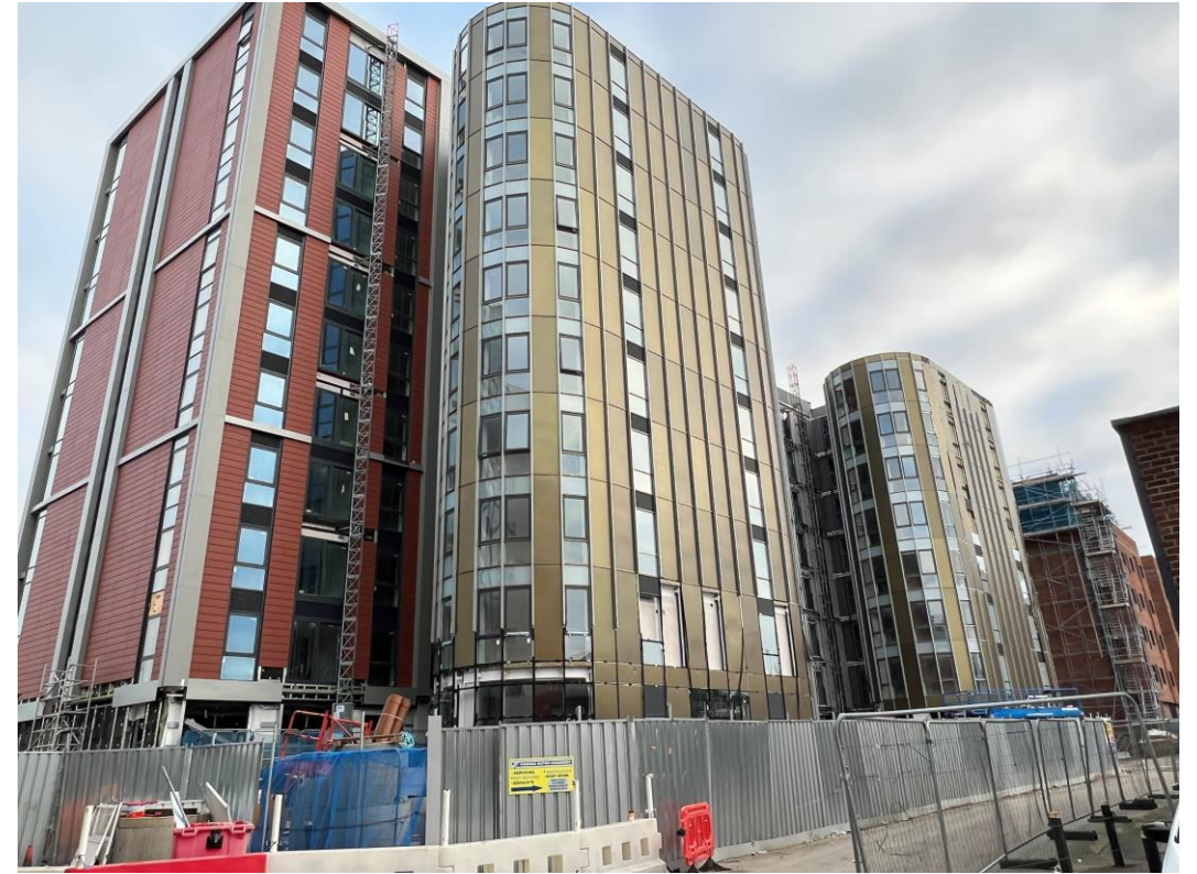
Caryl Street Elevation – cladding remedial works
