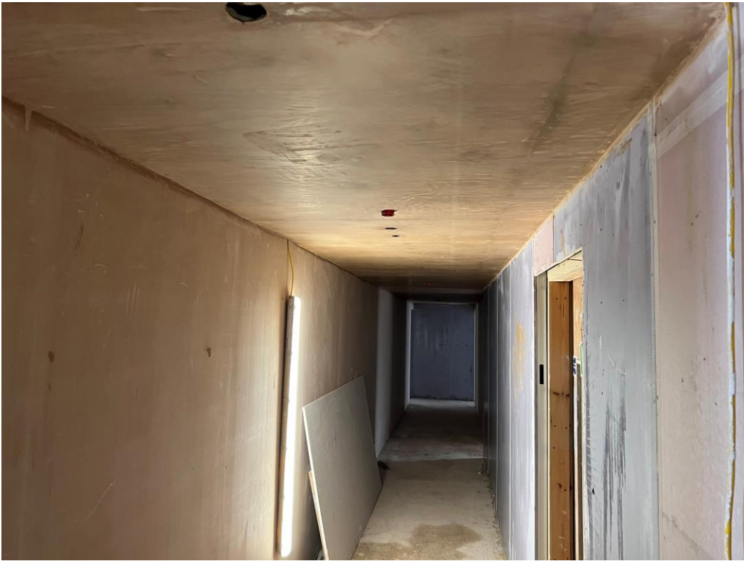
Block B – Ceilings skimmed to corridors
