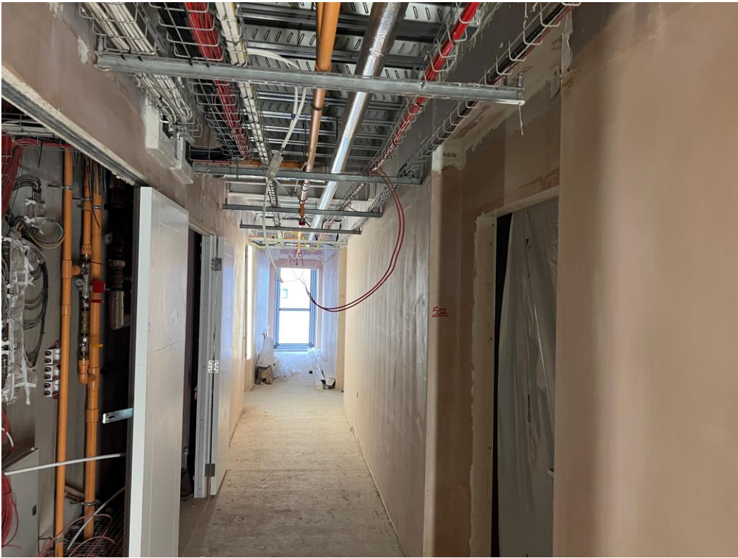
Block B – Walls skimmed to corridors
