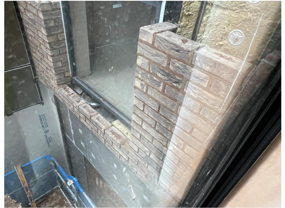
Brindley Steet Elevation – brickwork commenced
