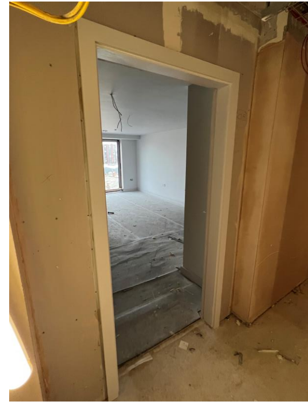
Architrave installed Apt door opening
