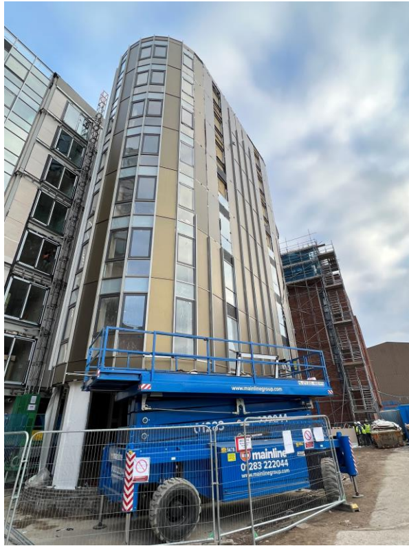
External cladding remedial works
