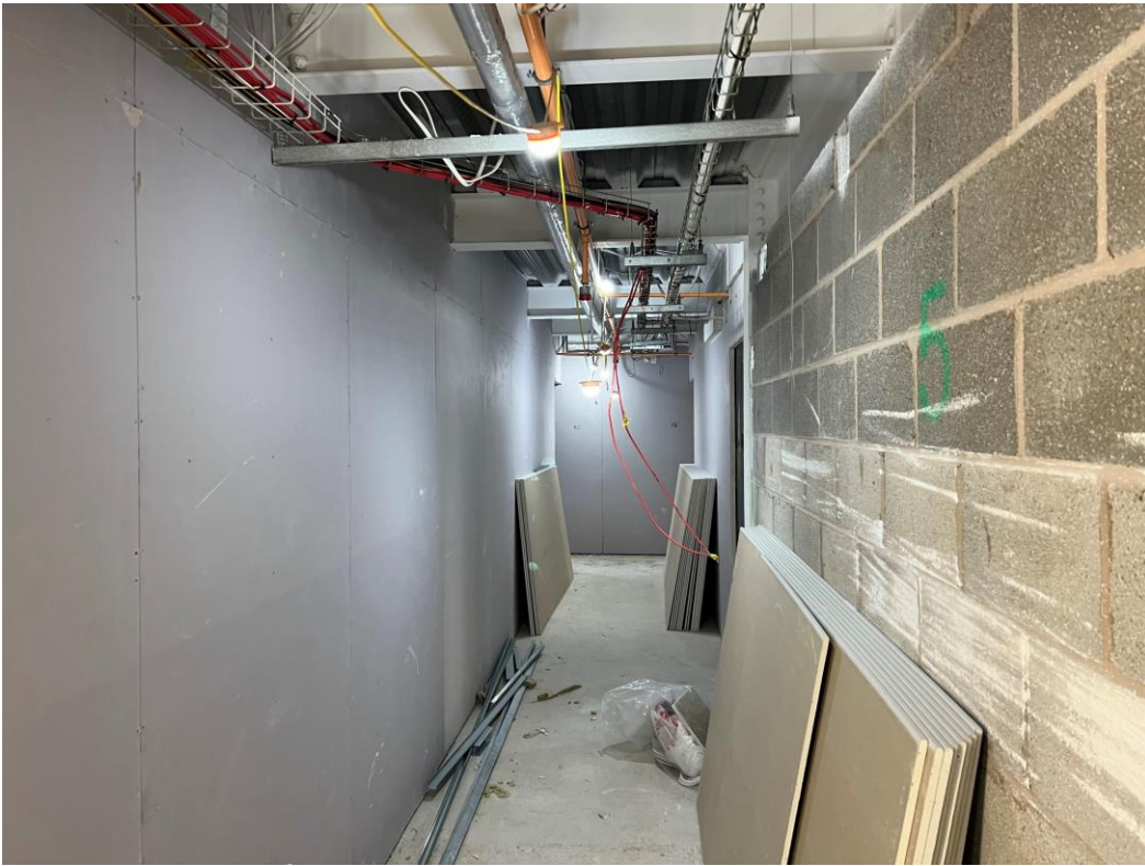
Block B – Wall boarding to corridors
