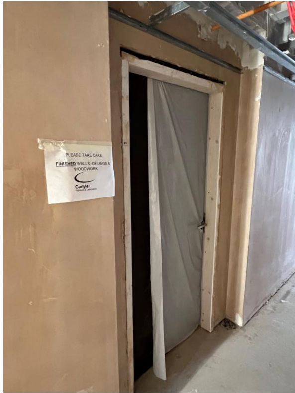
Apartment doors installed
