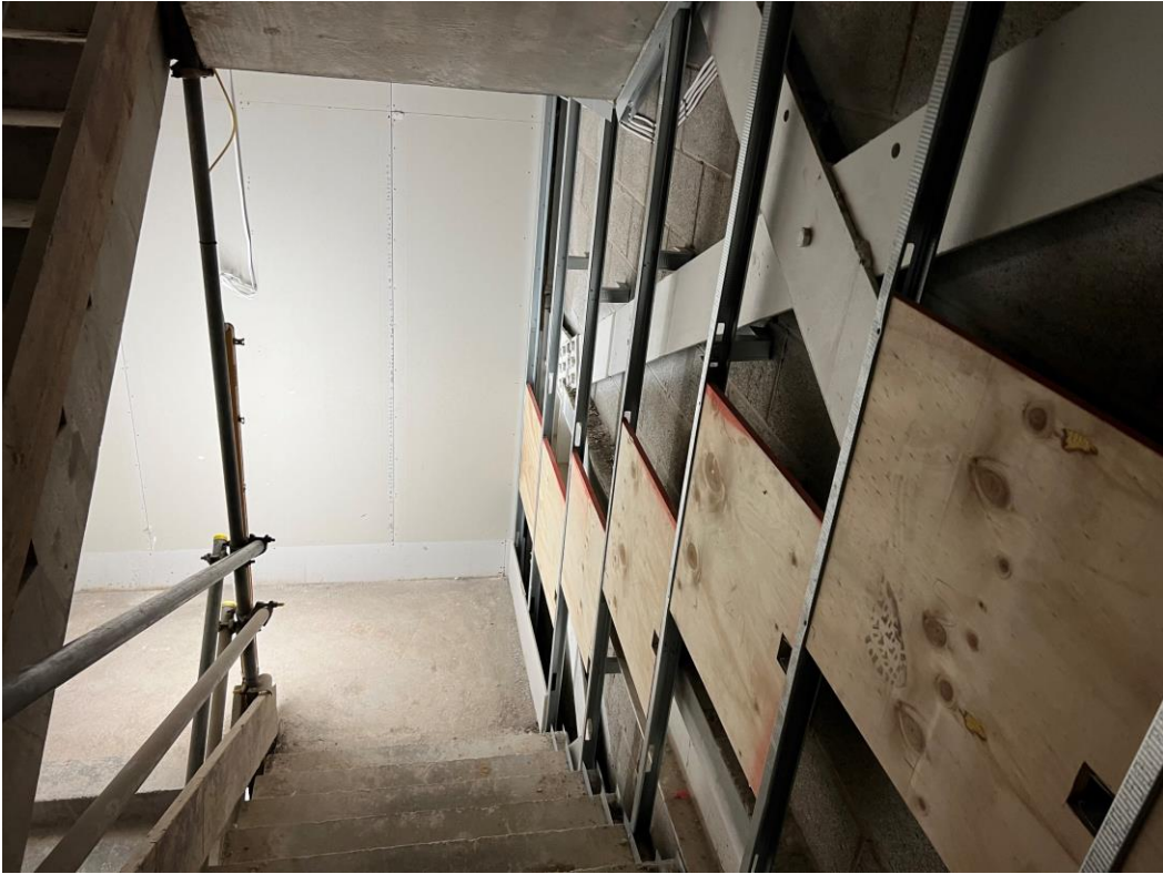
Partition & pattice installed to stairwell
