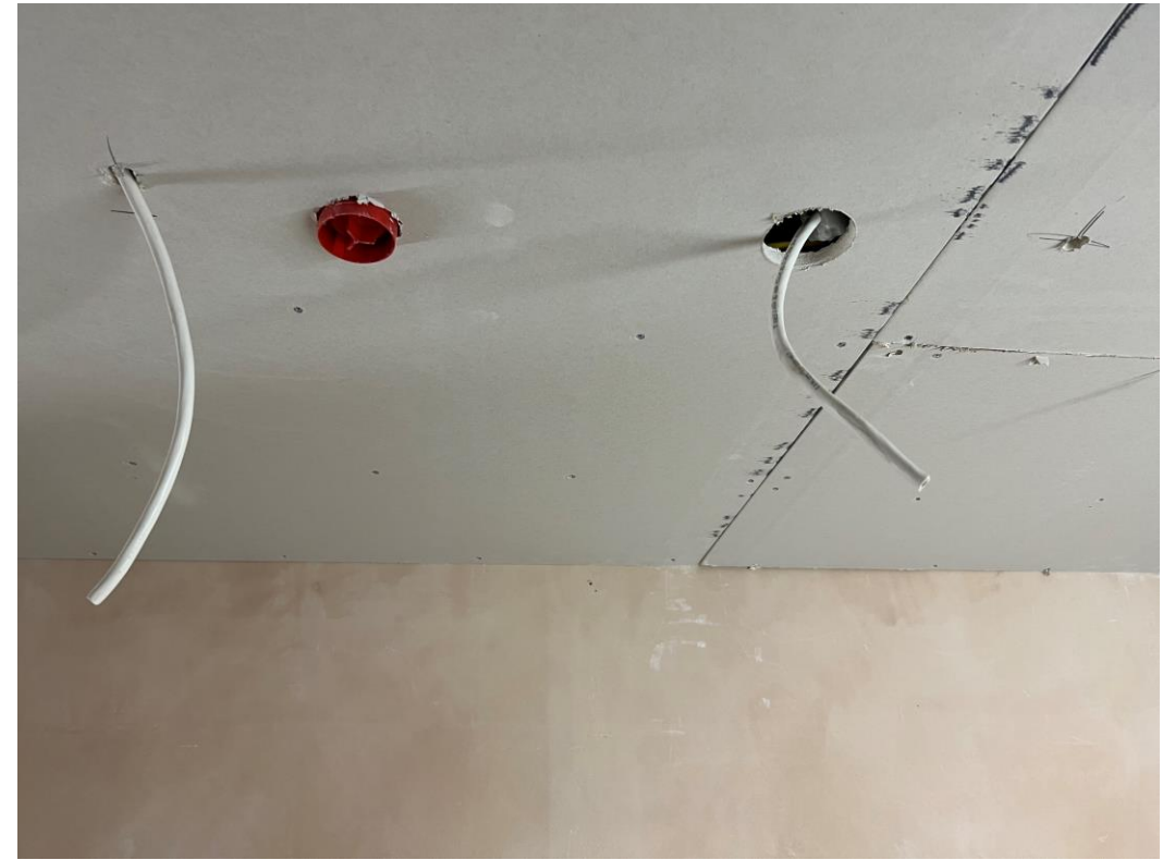
Electrical lighting installation commenced
