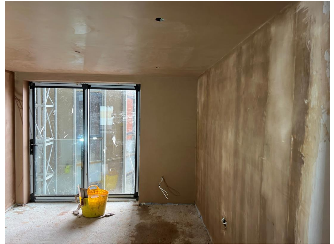
Walls & ceilings plaster skimmed to apartments
