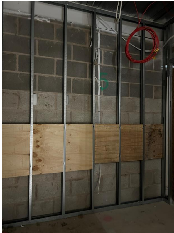
Partition & pattress installed to stairwell
