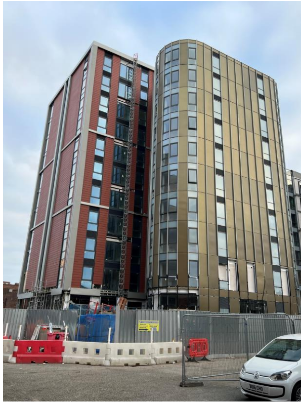
Caryl Street Elevation – cladding remedial works
