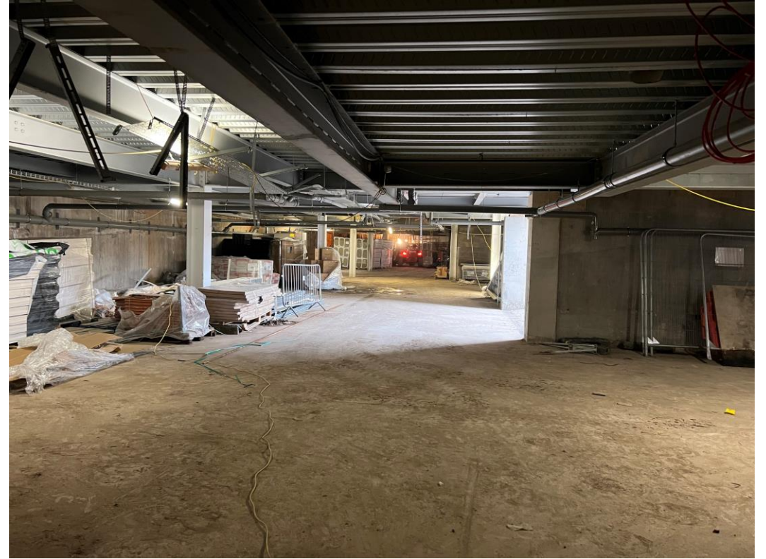
Basement site clearance ongoing
