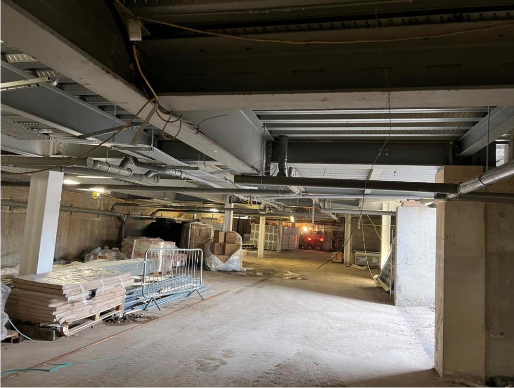
Basement site clearance ongoing
