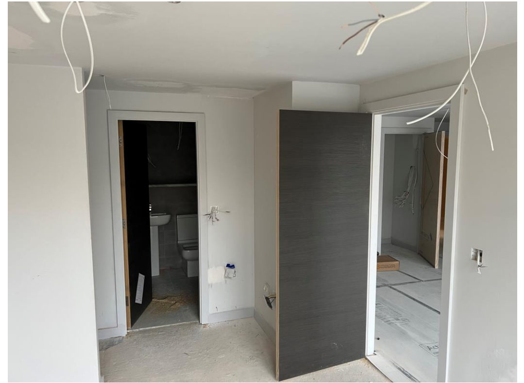
Apartment doors installed
