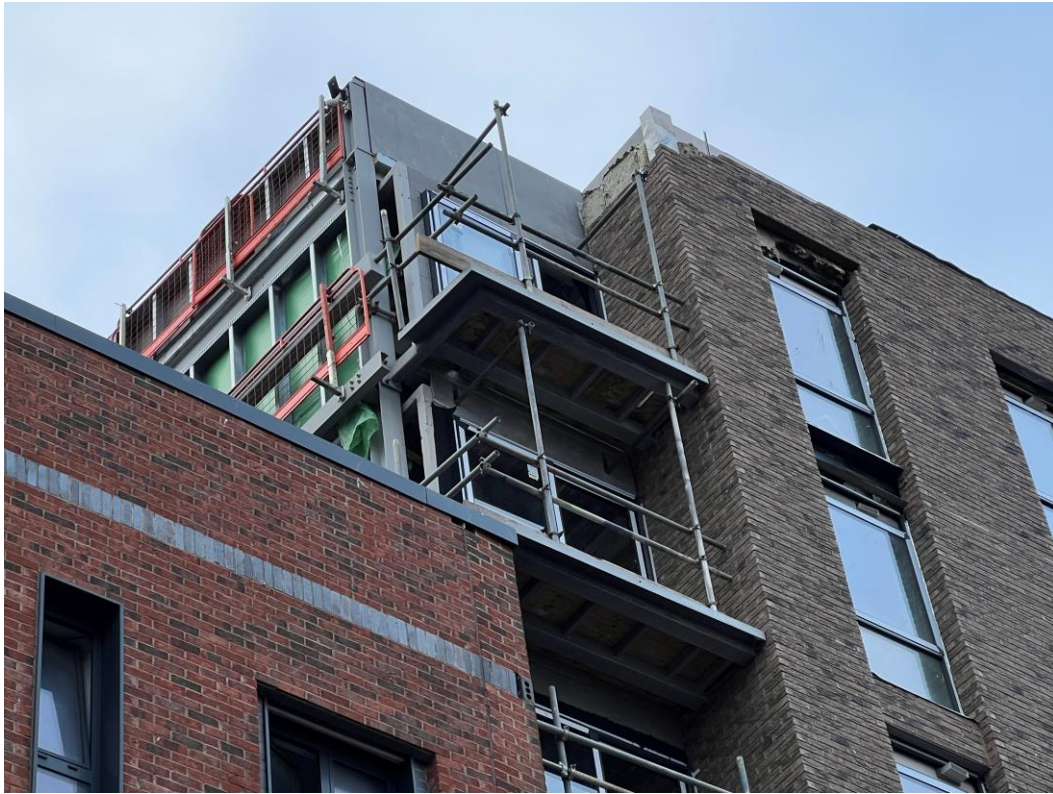
External cladding remedial works
