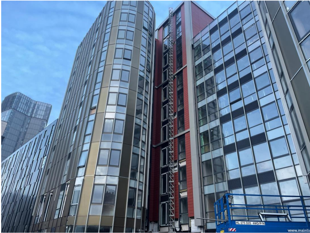
External cladding remedial works
