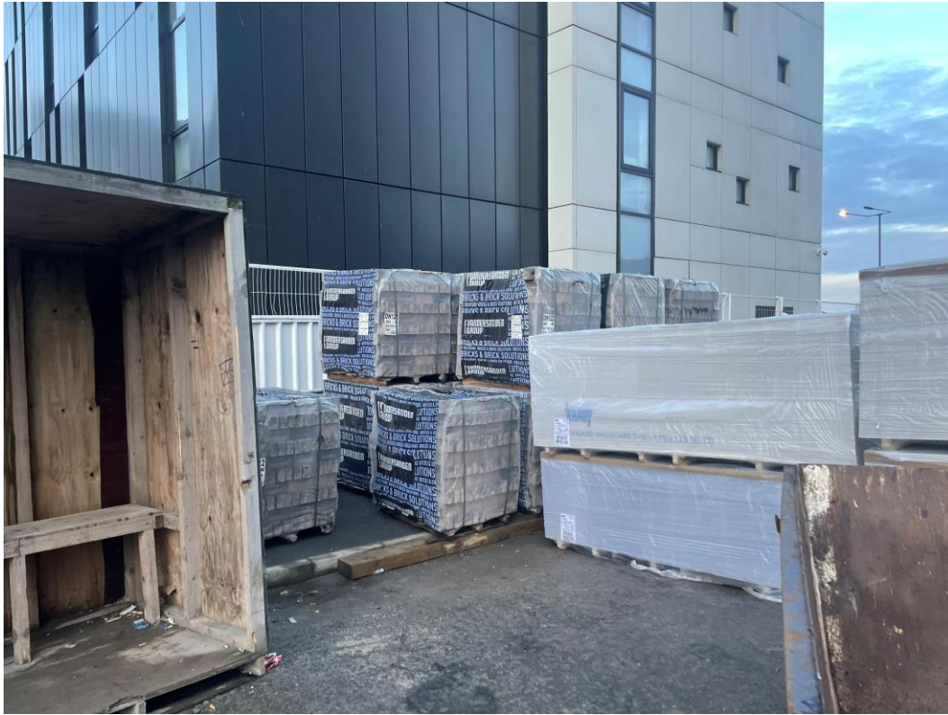
Brick & Plasterboard stored onsite
