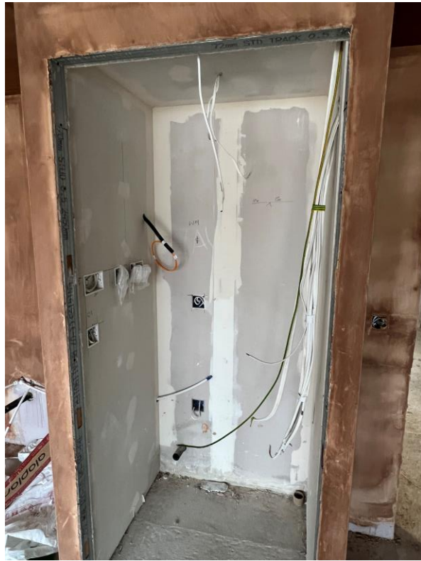
Walls & ceilings plaster skimmed to apartments
