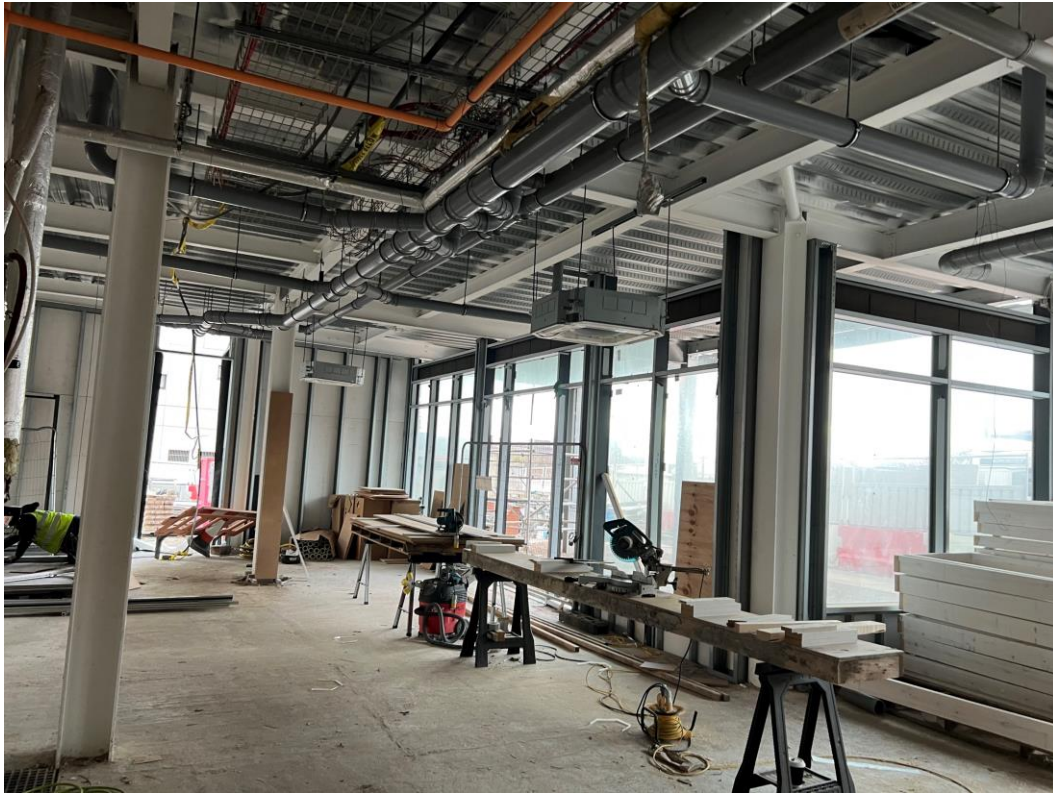
Ground floor site activity
