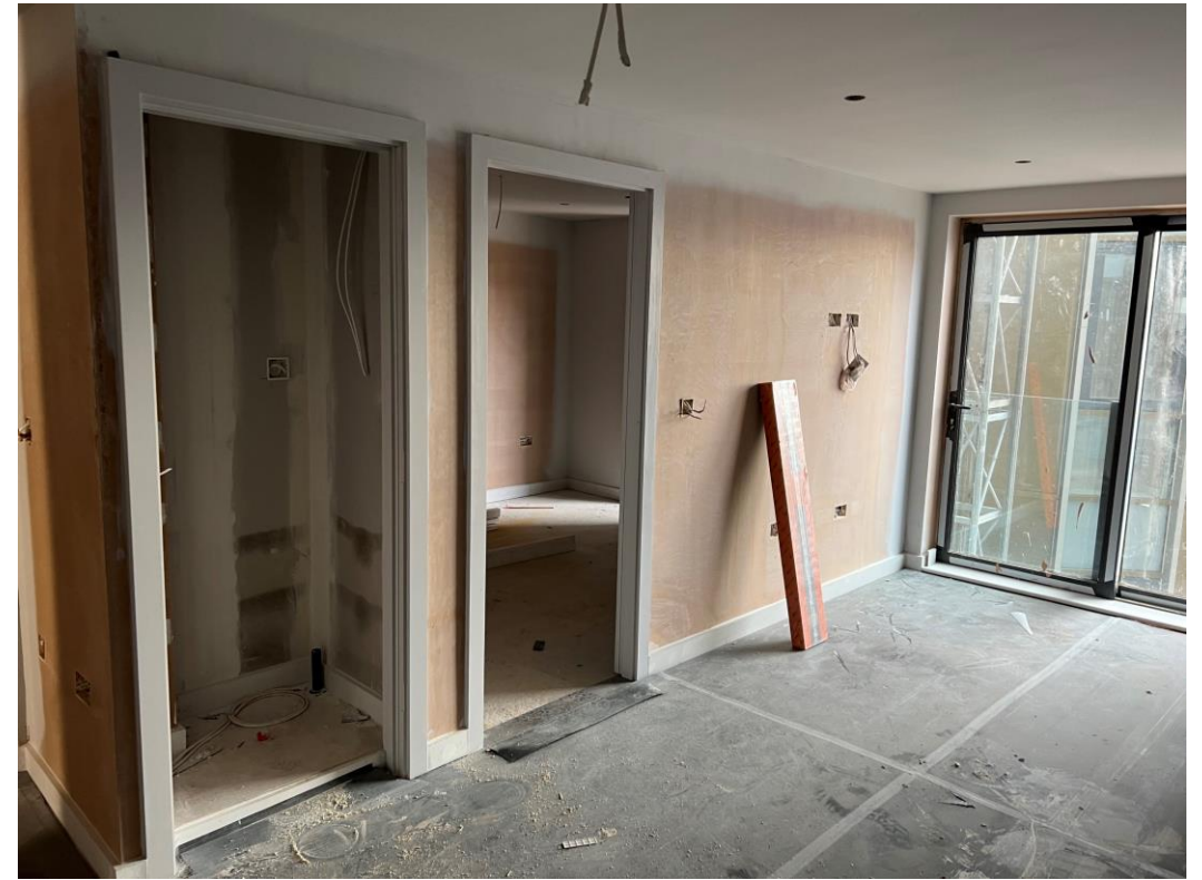
Skirting Boards & Architraves installed
