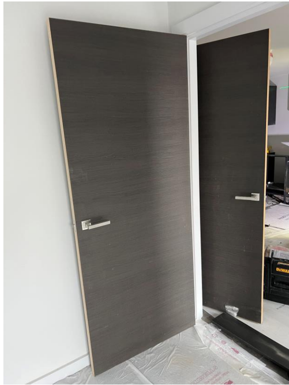
Apartment doors installed
