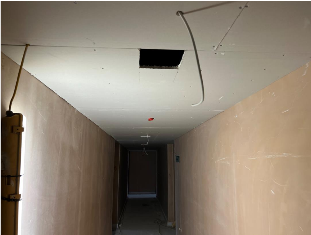
Block B – Ceilings boarded to corridors
