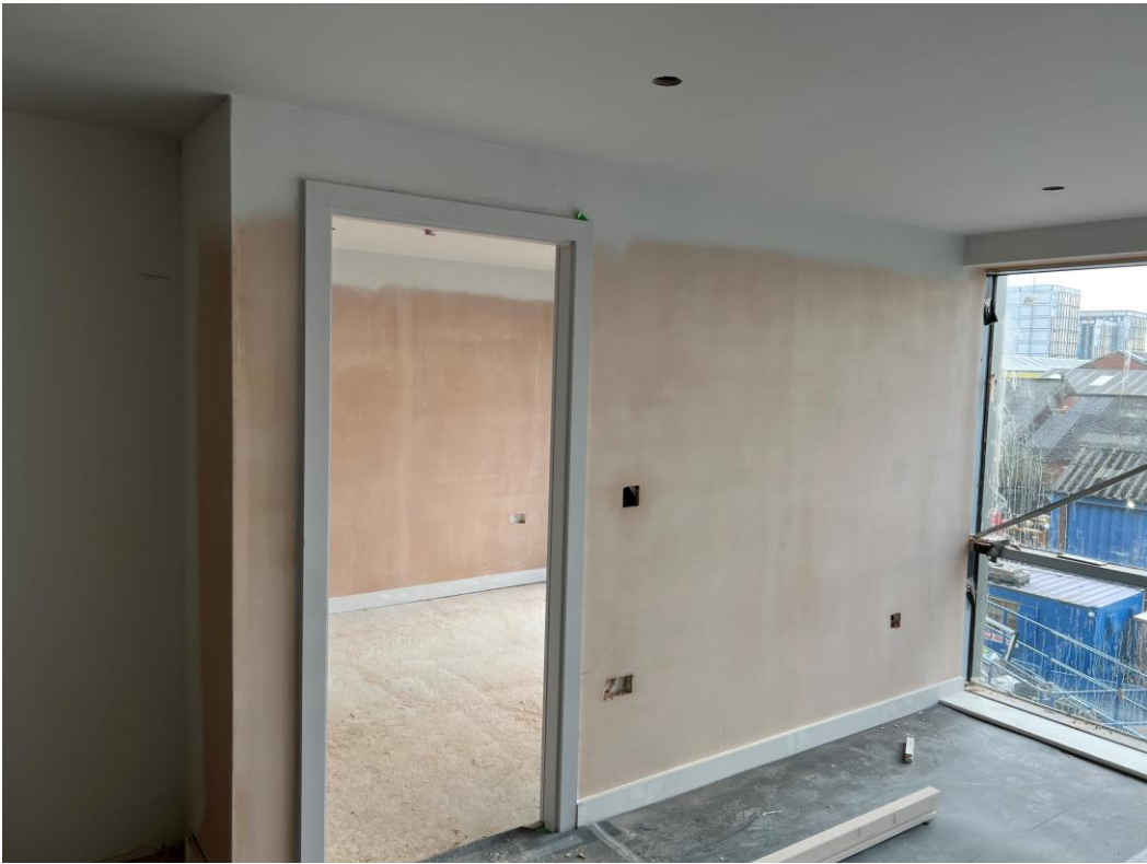
Skirting Boards & Architraves installed
