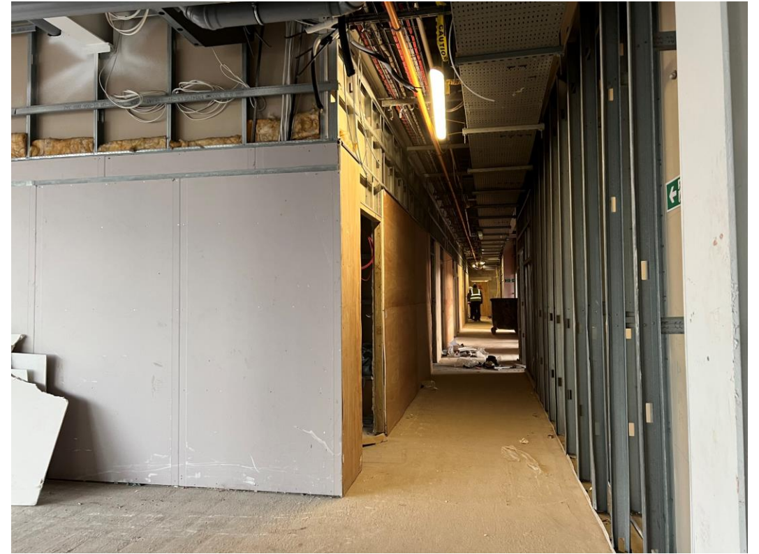
Ground floor site activity
