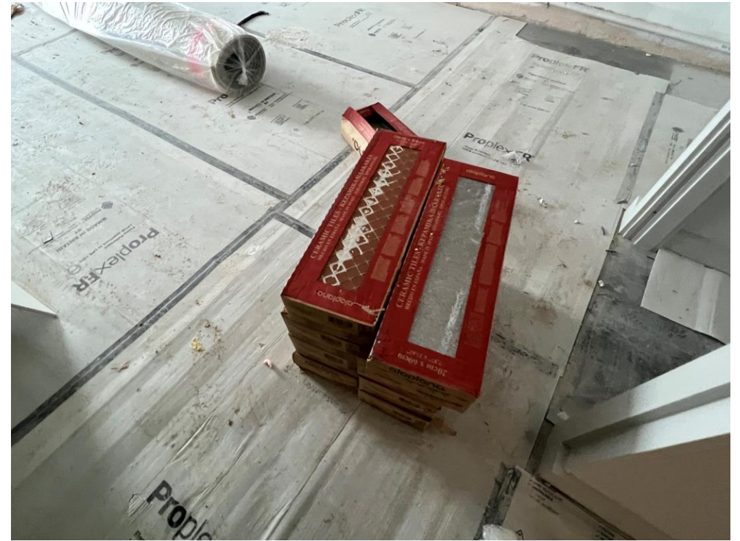
Bathroom wall tiles loaded for installation
