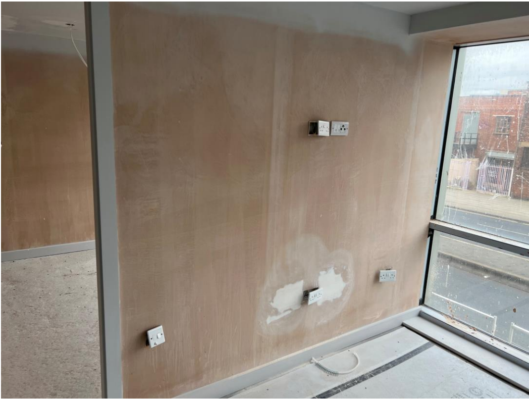
2 nd Fix electrics to feature wall
