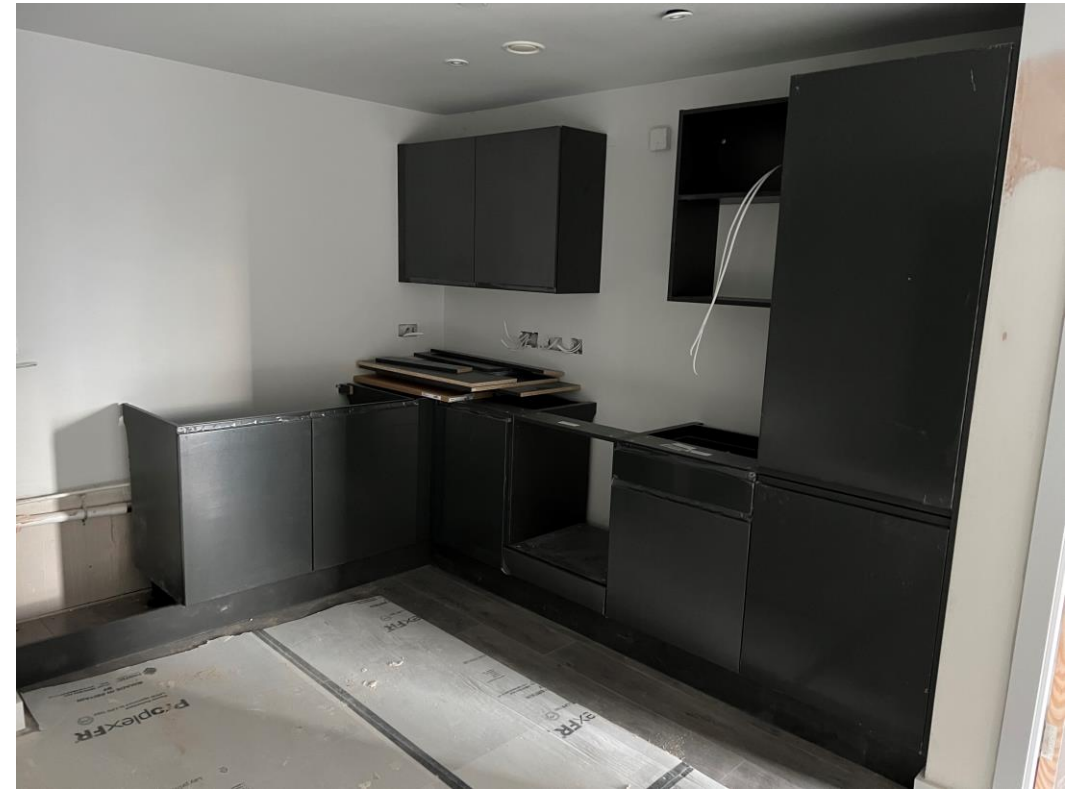
Block A – Kitchen units commenced
