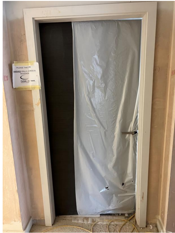
Apartment doors installed
