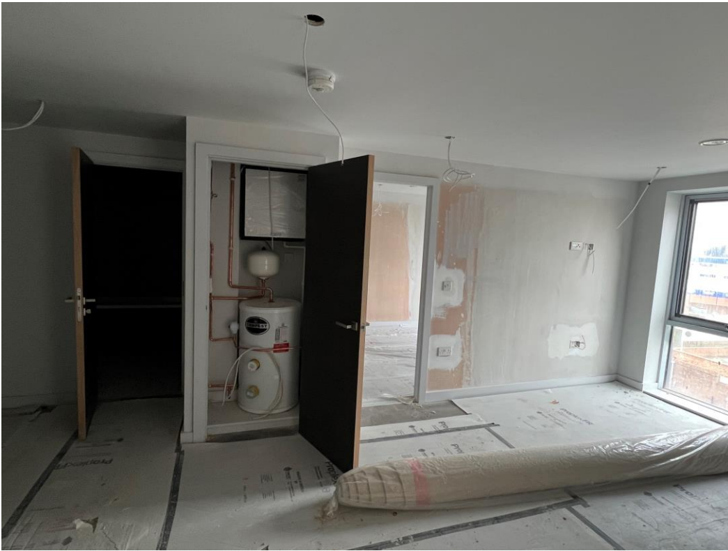
Apartment doors installed
