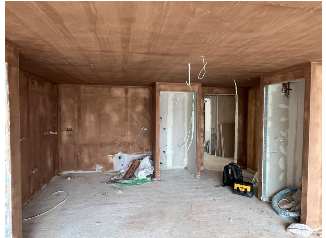
Apartment walls & ceilings plaster skimmed
