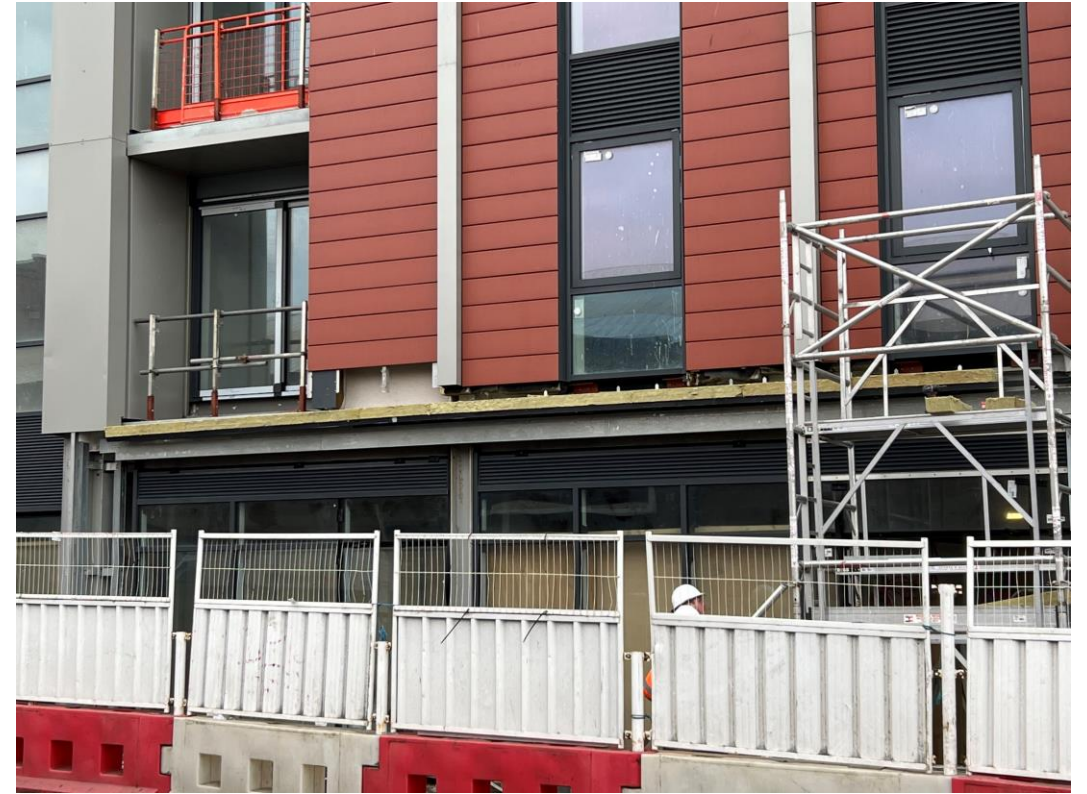
Cladding remedial works to Parliament Street Elevation
