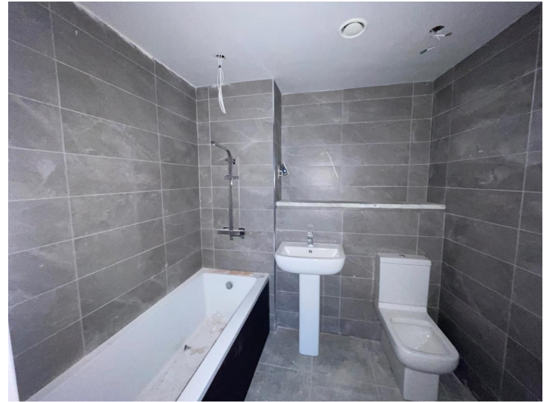
Bathroom installation ongoing
