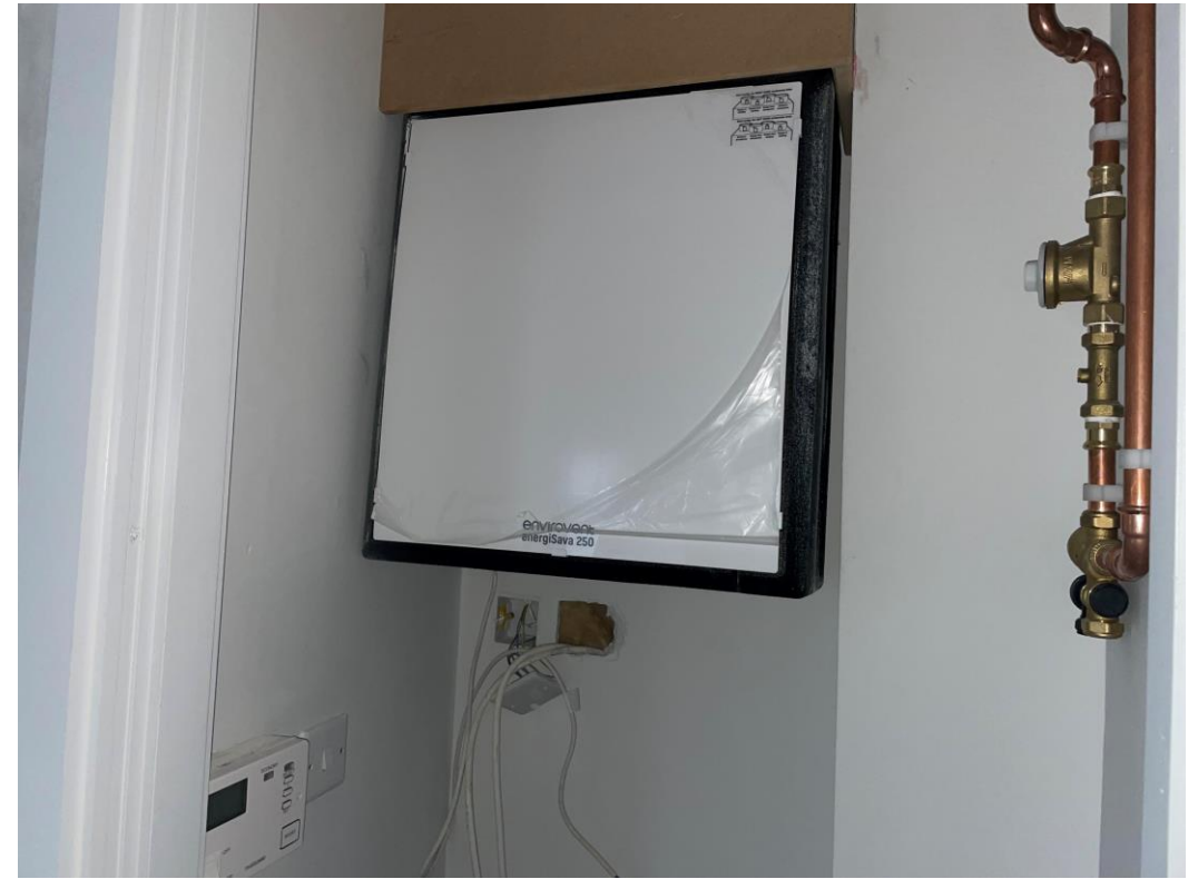
Ventilation system installation ongoing
