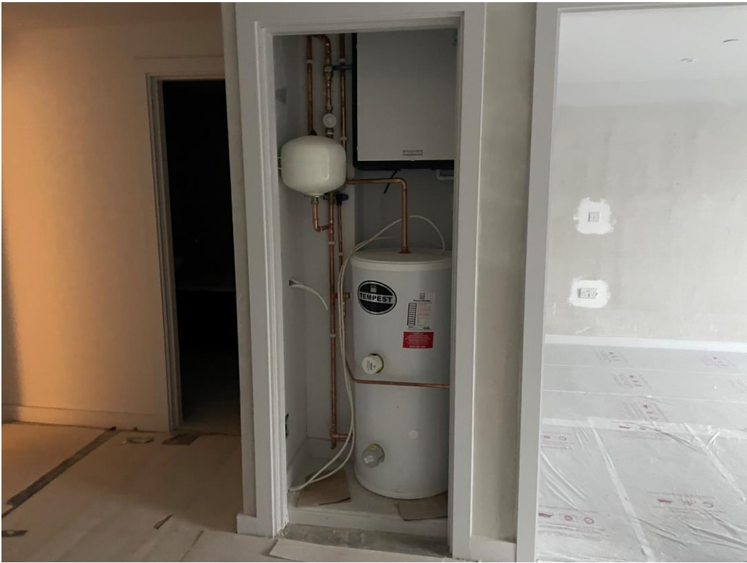
Ventilation system & water cylinder installation ongoing
