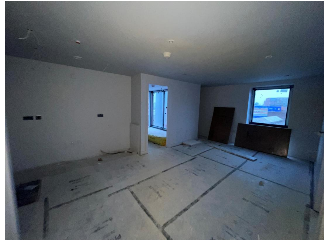
Decoration ongoing to apartments
