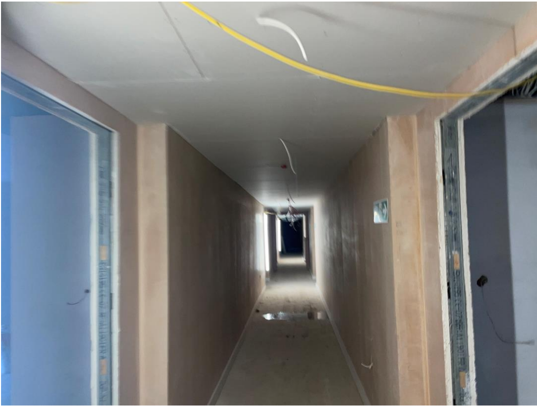
Ceilings boarded to circulation areas
