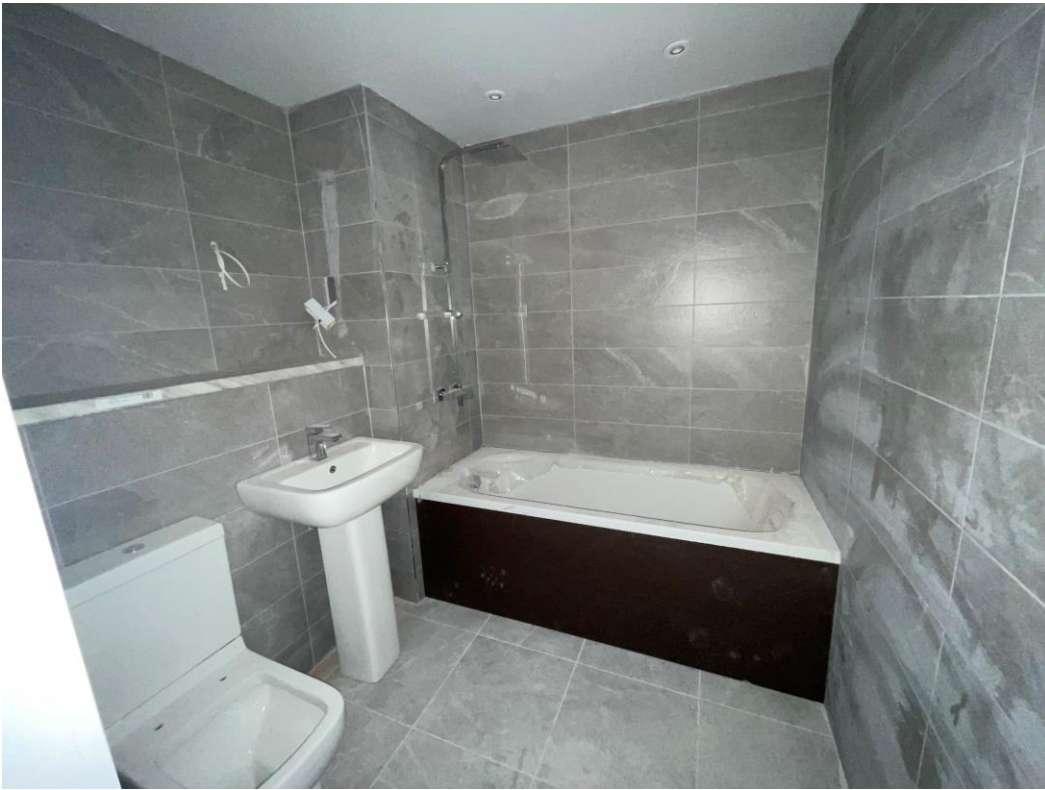
Bathroom installation nearing completion
