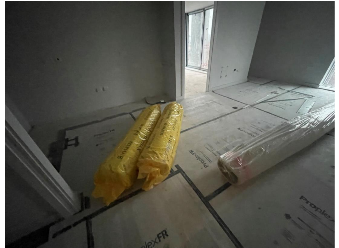
Carpets & underlay on site ready for installation
