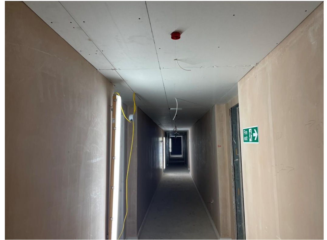
Ceilings boarded & walls skimmed to circulation areas
