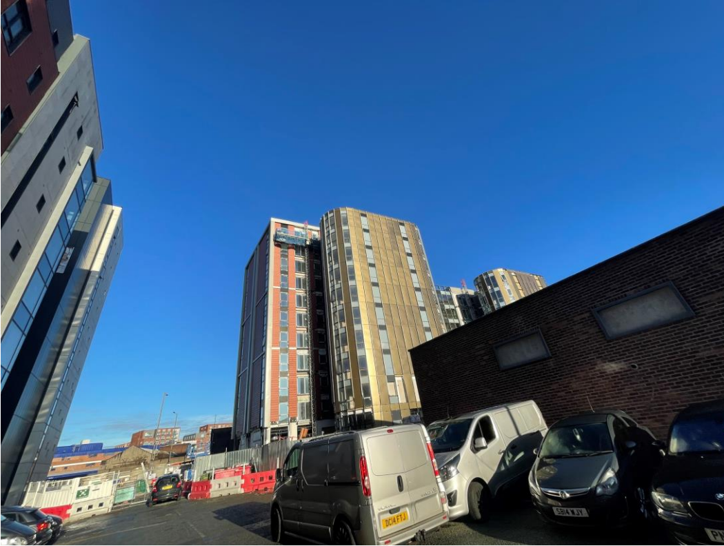
Development viewed from Caryl Street
