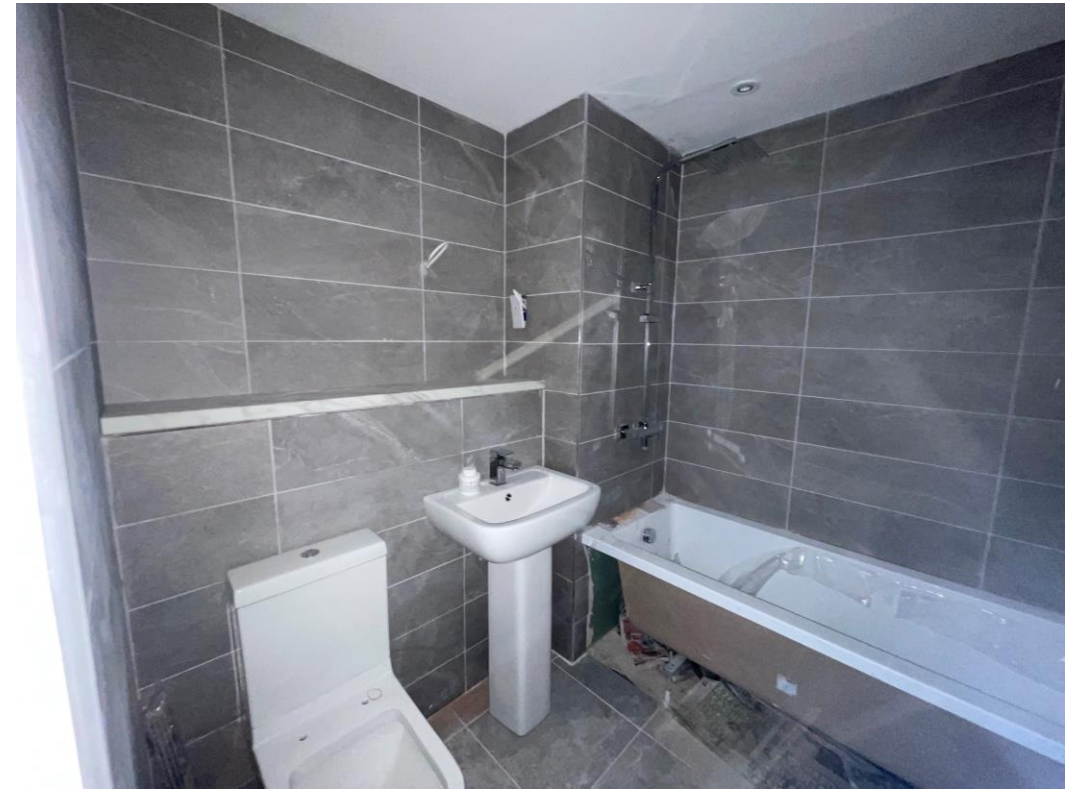
Sanitary & vanity shelf installation ongoing
