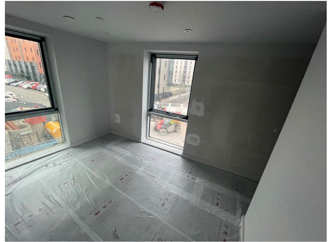
Carpets installation ongoing
