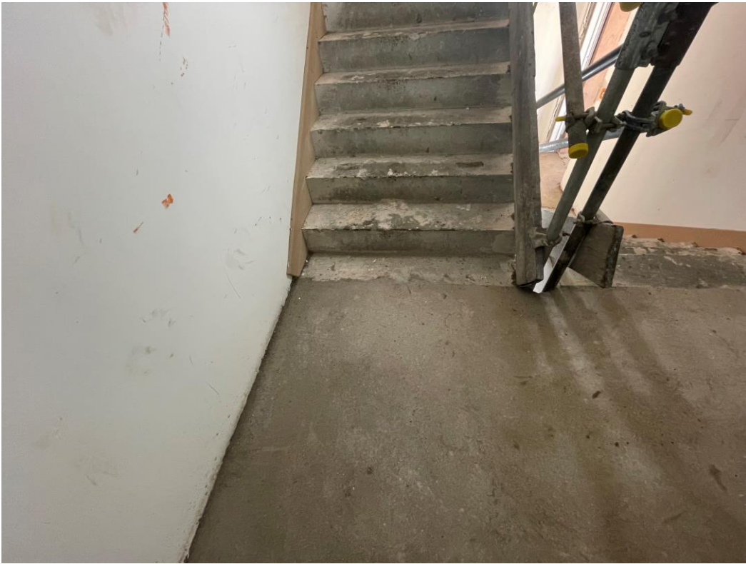
Screeding to landing areas ongoing
