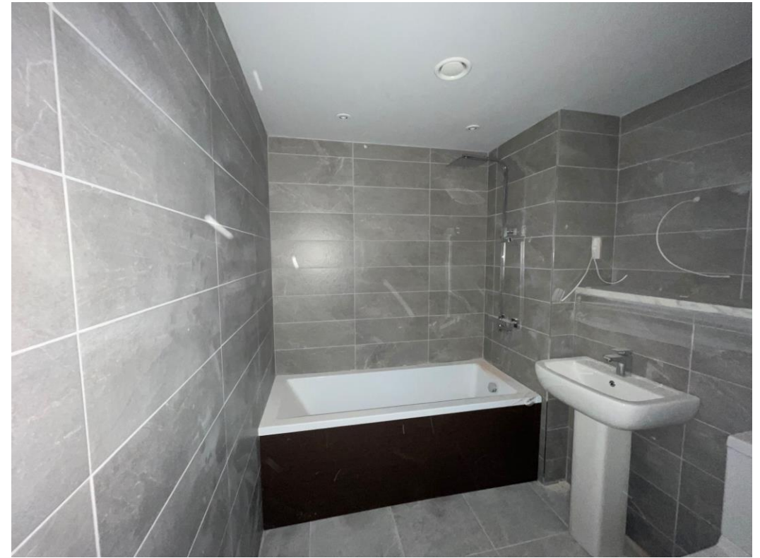
Bath panel installed
