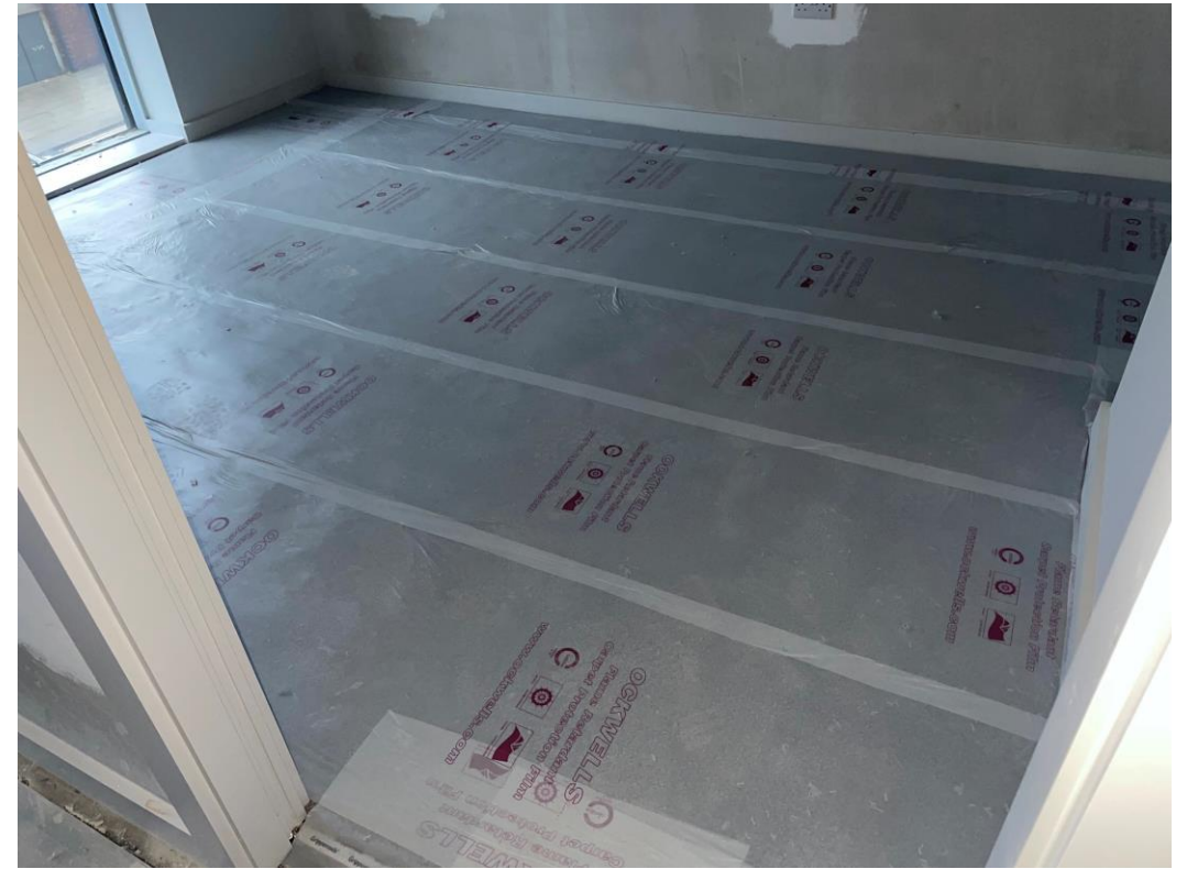
Carpets installation ongoing
