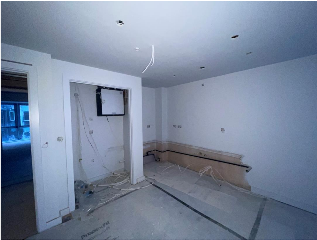
Ventilation system installation ongoing
