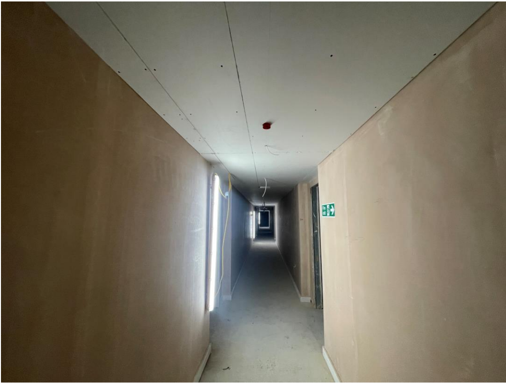
Ceilings boarded & walls skimmed to circulation areas
