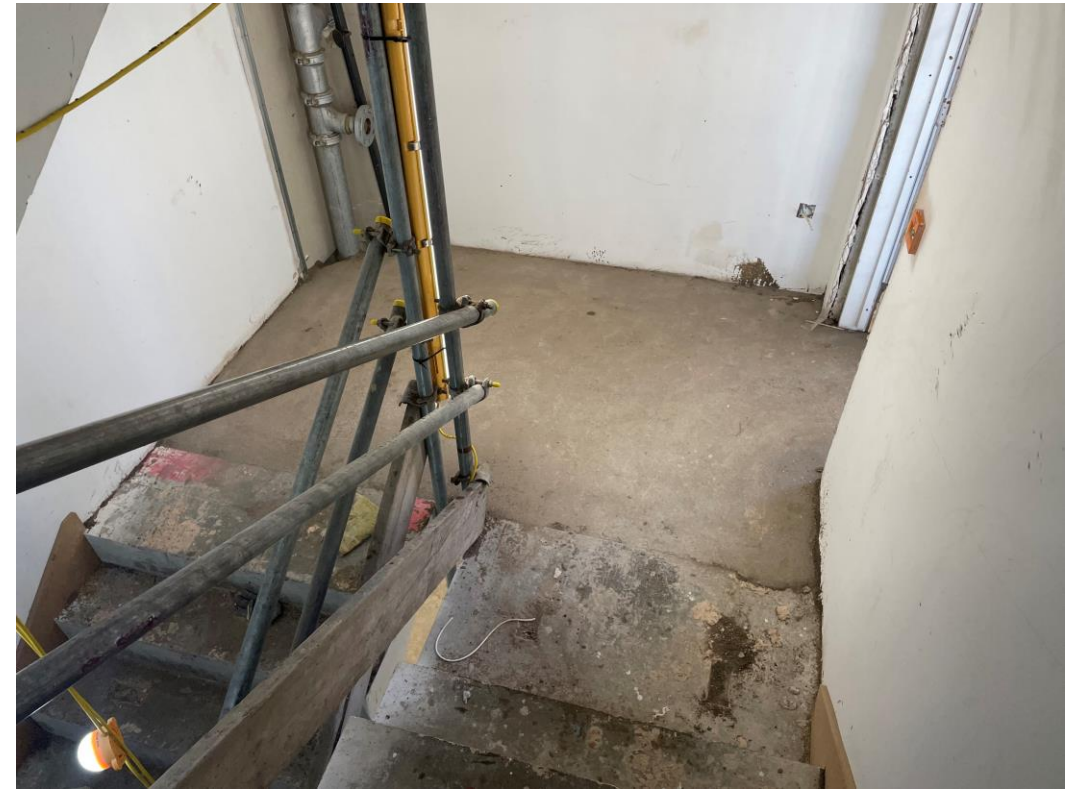
Screeding to landing areas ongoing
