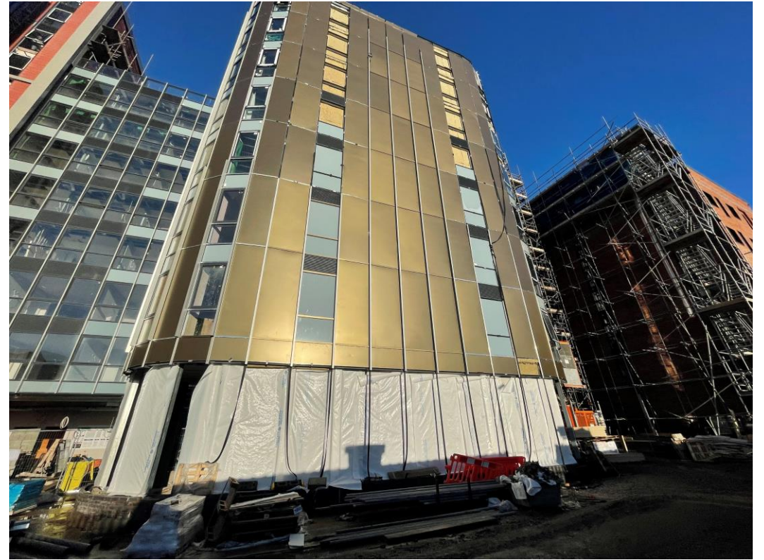
Curtain walling installation to ground floor ongoing
