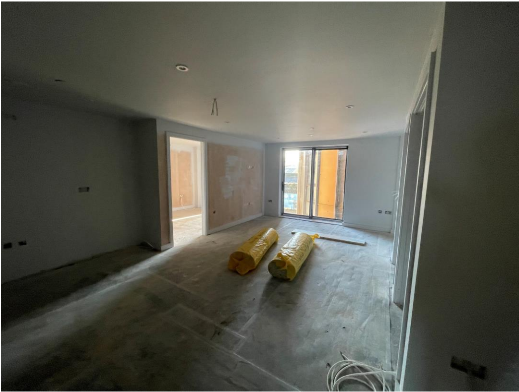
Carpets onsite ready for installation
