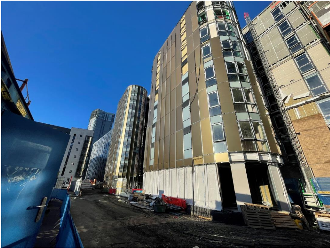
Curtain walling installation to ground floor ongoing
