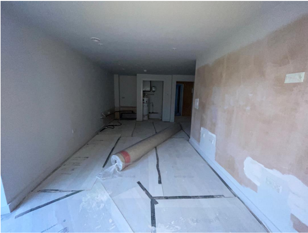
Carpets & underlay on site ready for installation
