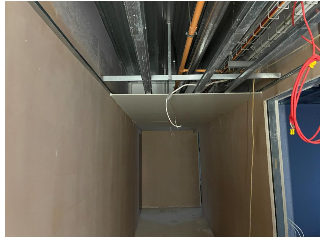
Ceiling grid installed & walls skimmed to circulation areas
