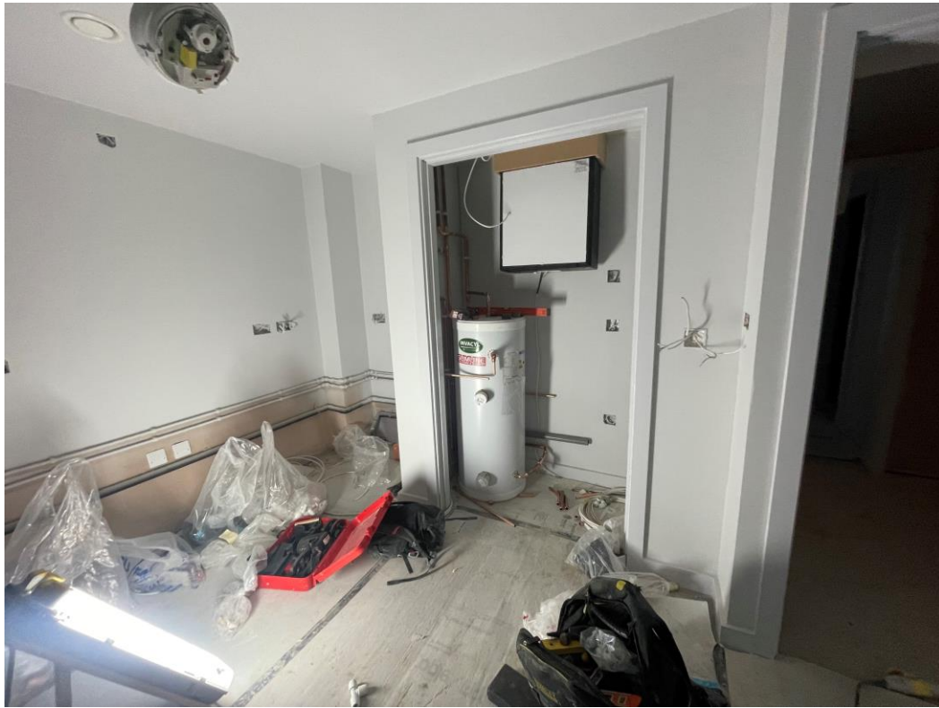
Ventilation system & water cylinder installation ongoing
