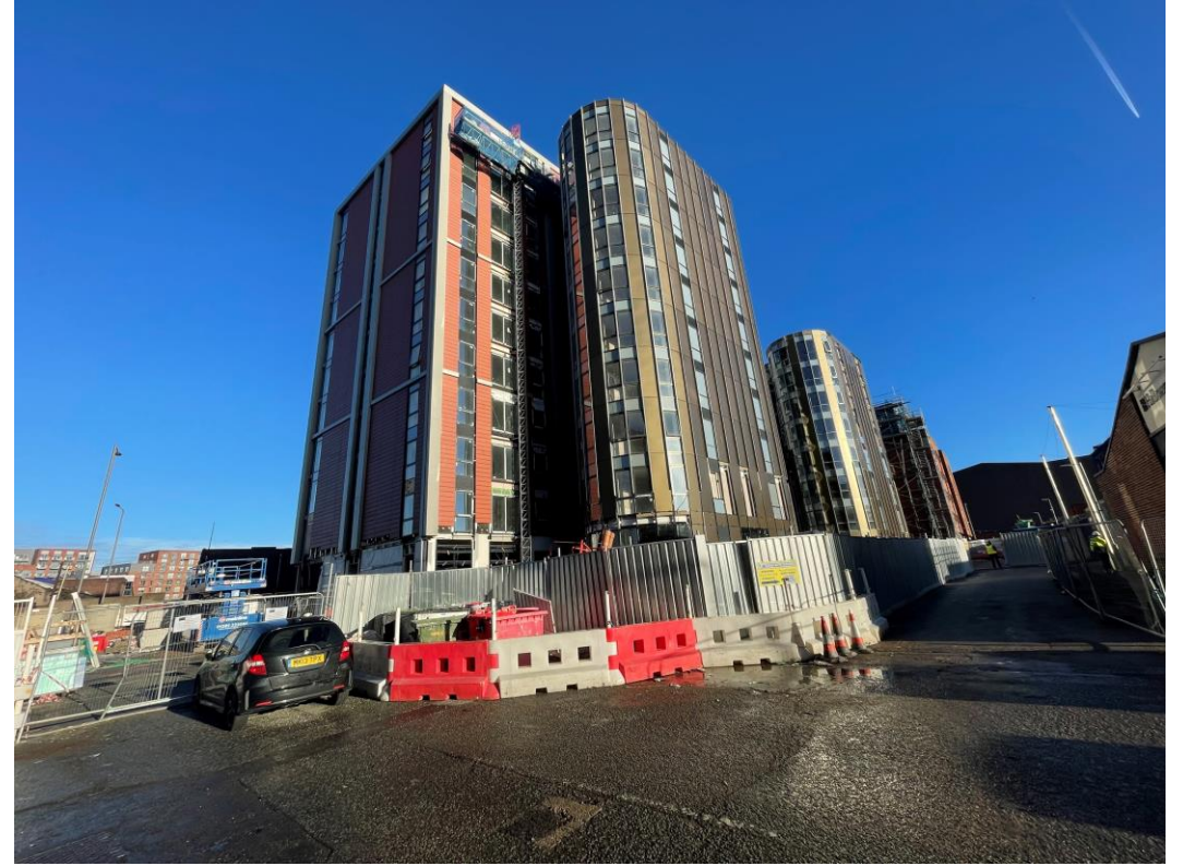
External Cladding remedial works ongoing
