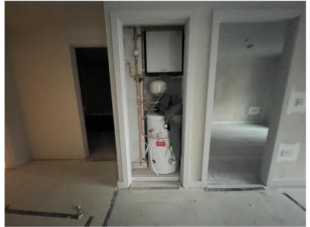
Ventilation system & water cylinder installation ongoing
