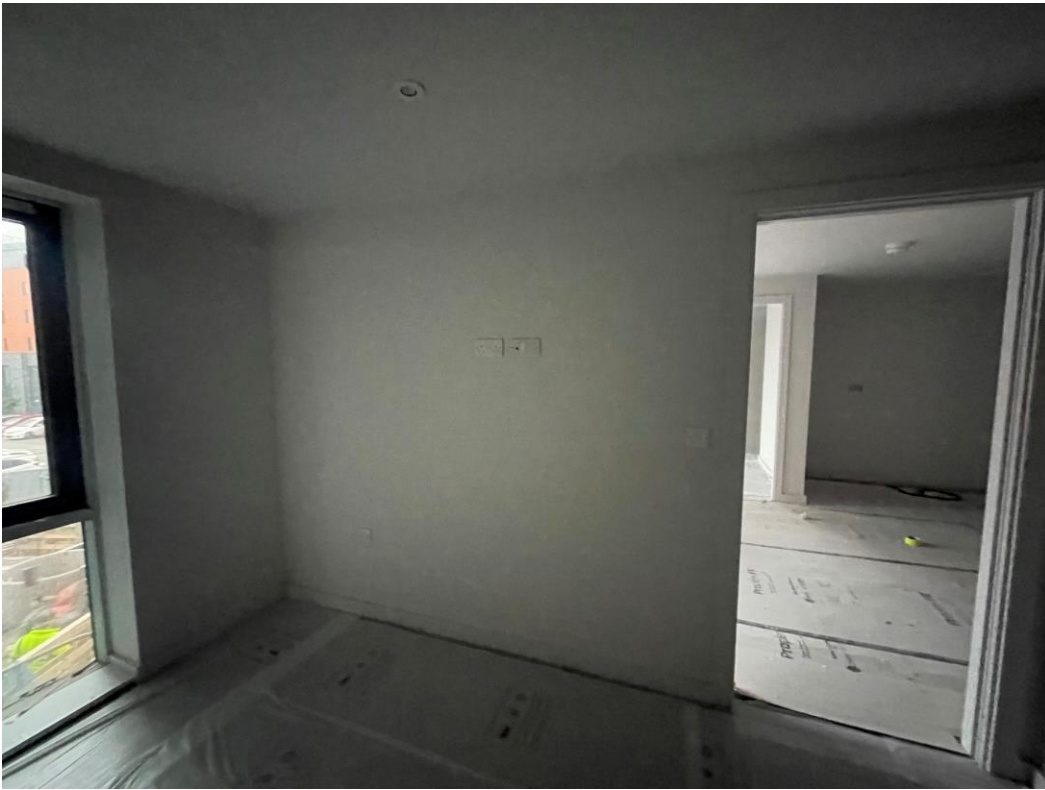
Carpets installation ongoing
