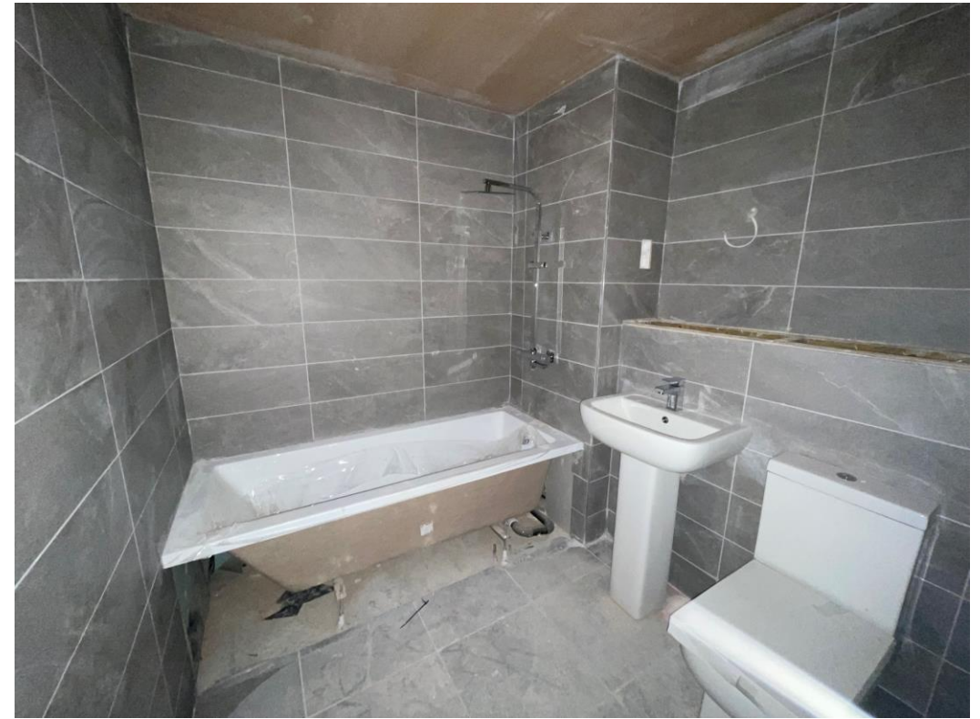
Bath & shower installed
