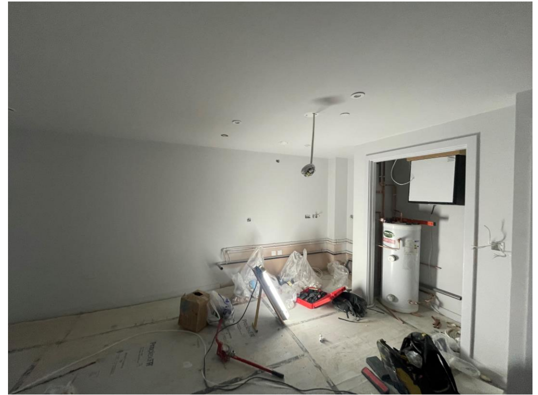
Ventilation system & water cylinder installation ongoing
