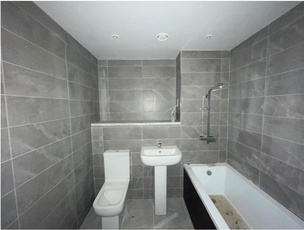
Bathroom installation nearing completion
