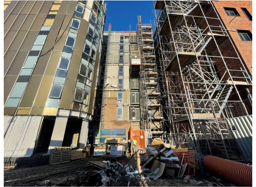
Curtain walling installation to ground floor ongoing
