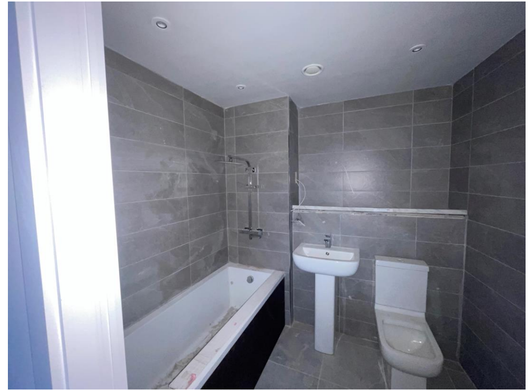
Bathroom installation ongoing
