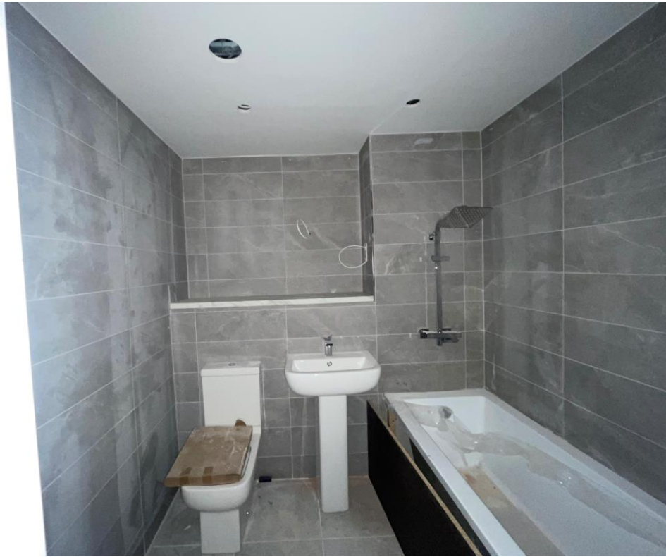
Bathroom installation ongoing
