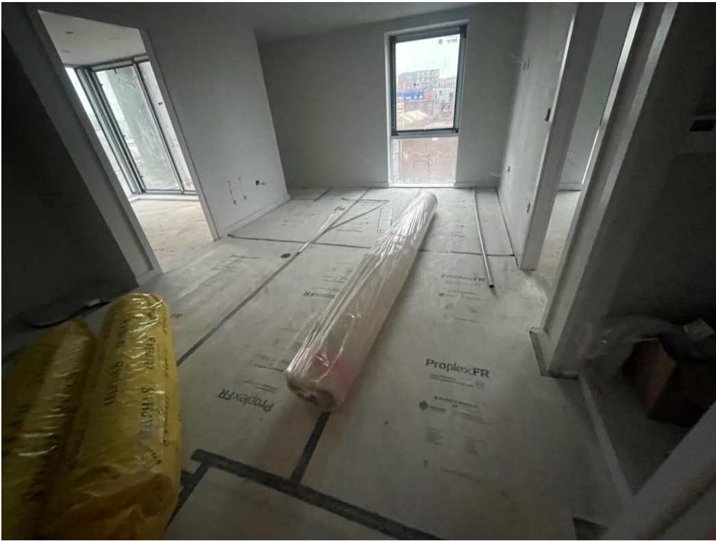
Carpets onsite ready for installation
