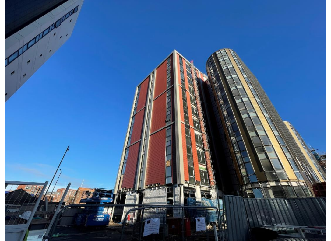
Development viewed from Caryl Street
