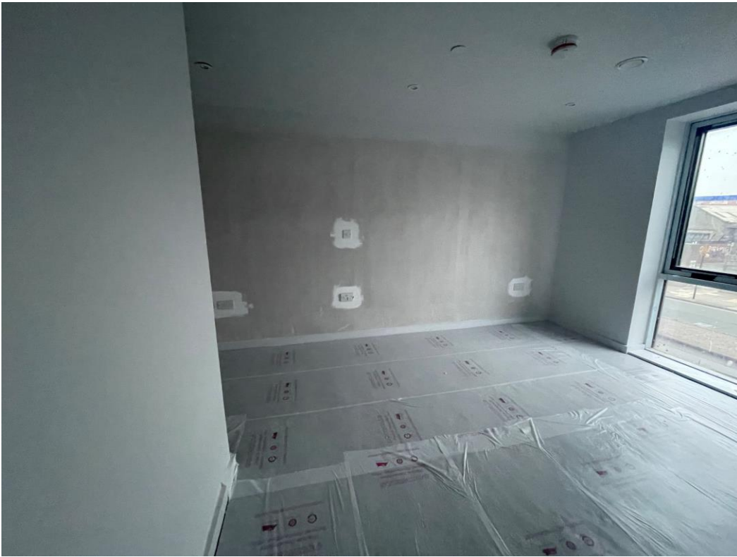
Carpet installation ongoing
