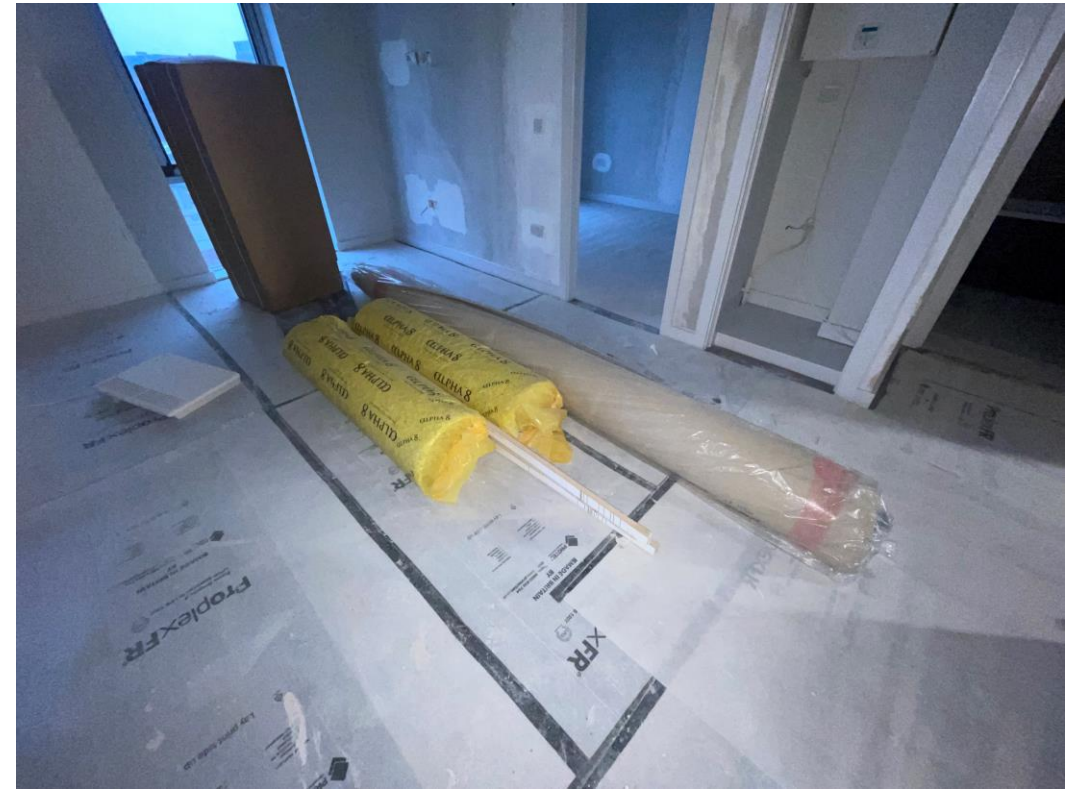
Carpets & underlay on site ready for installation
