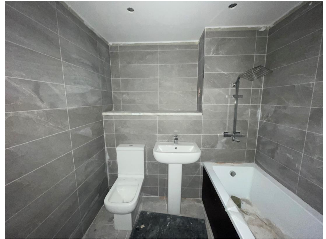
Sanitary & vanity shelf installation ongoing
