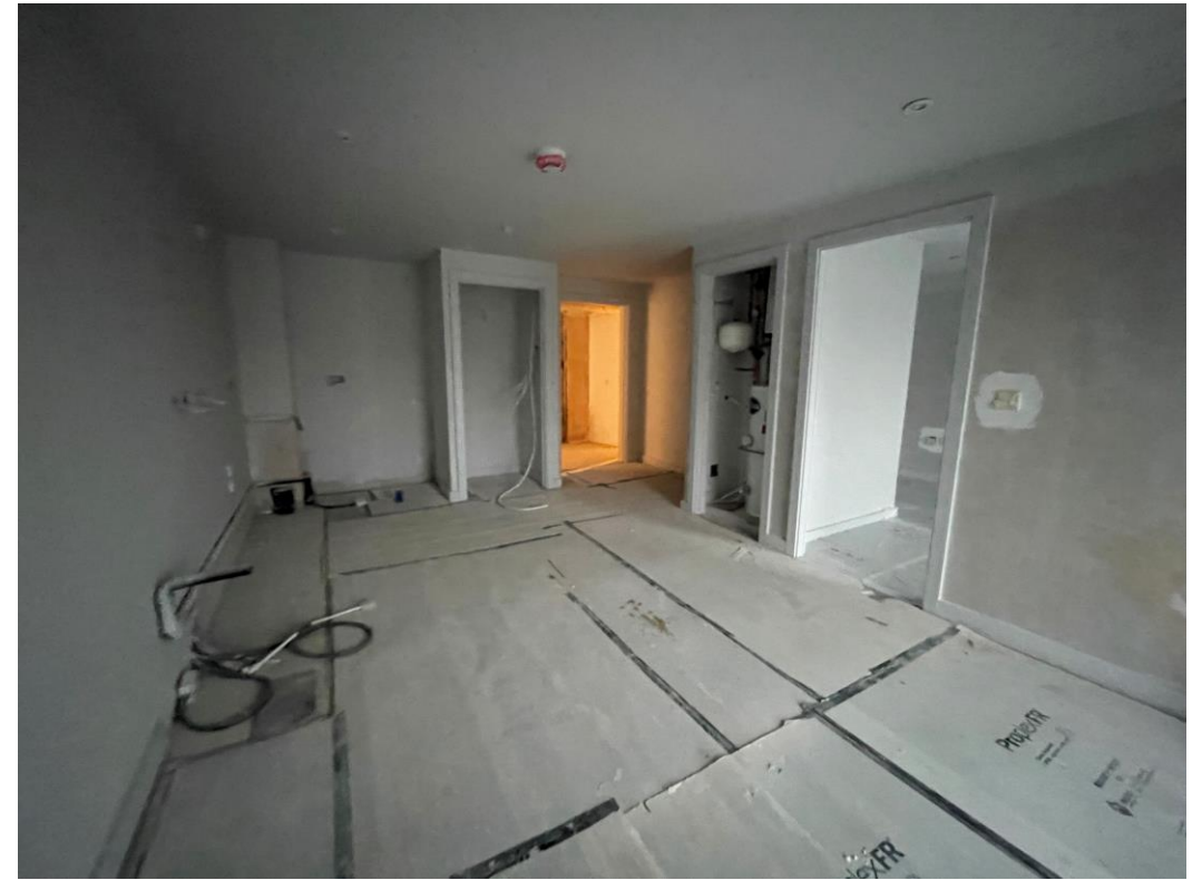
Decoration ongoing to apartments
