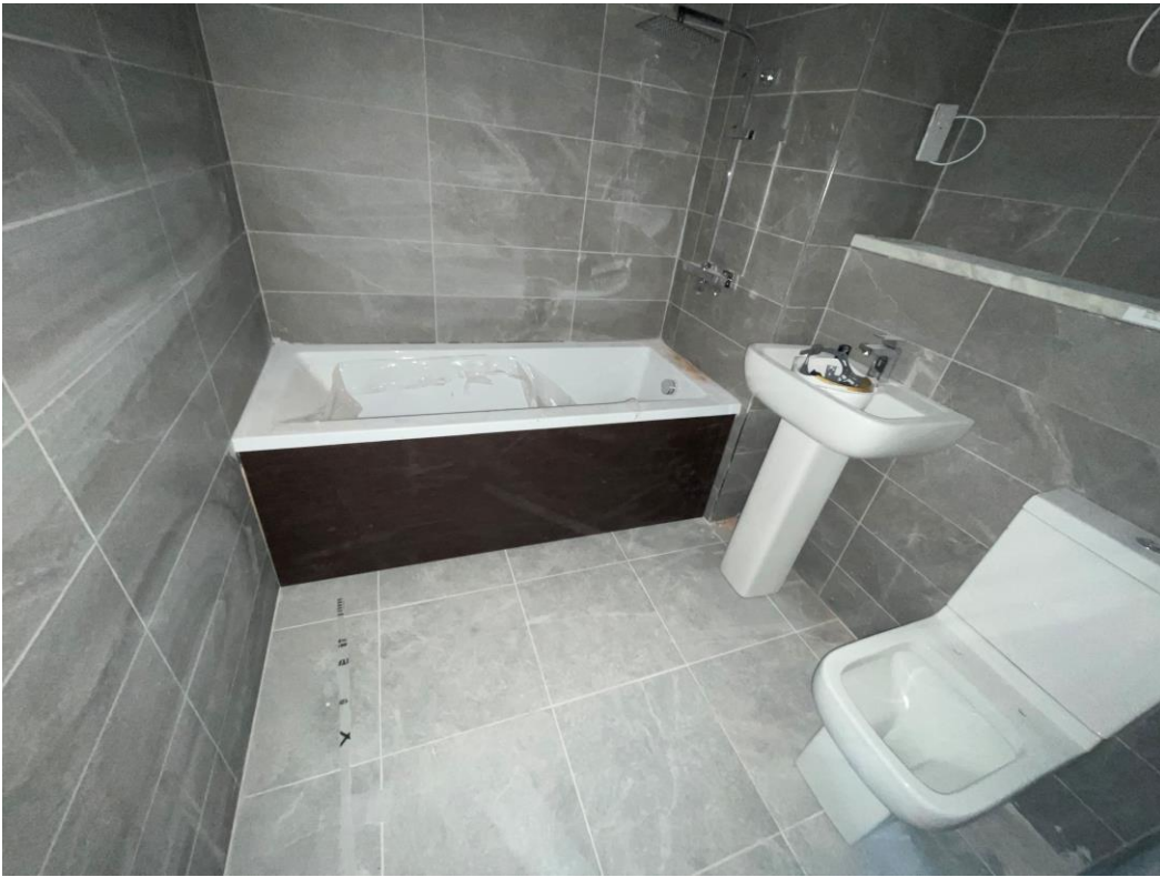
Sanitary & vanity shelf installation ongoing
