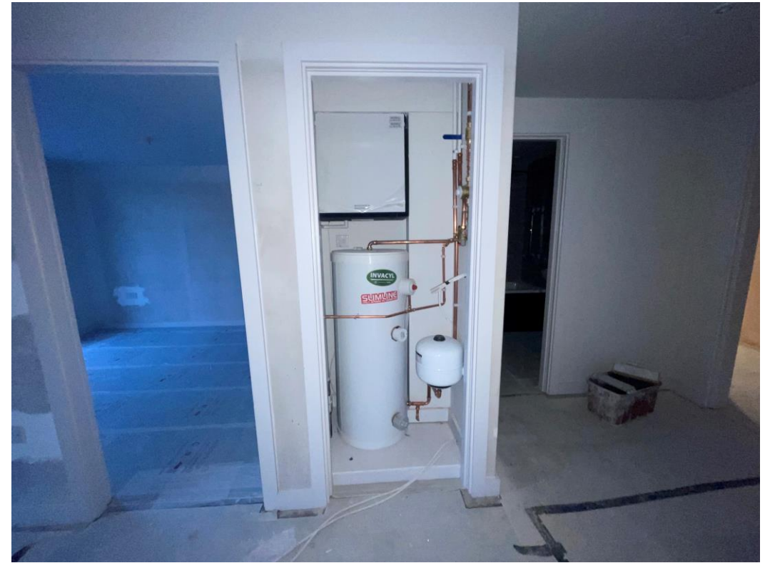
Ventilation system & water cylinder installation ongoing
