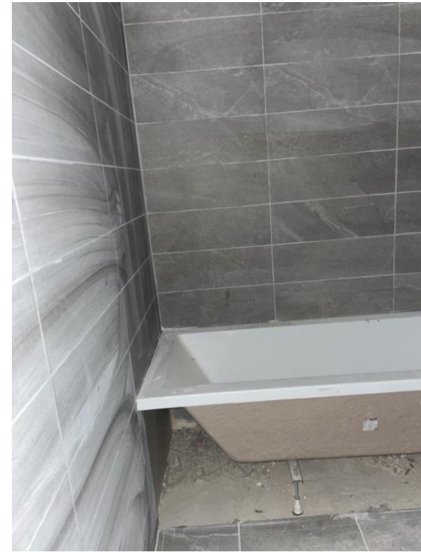
Sanitary installation ongoing
