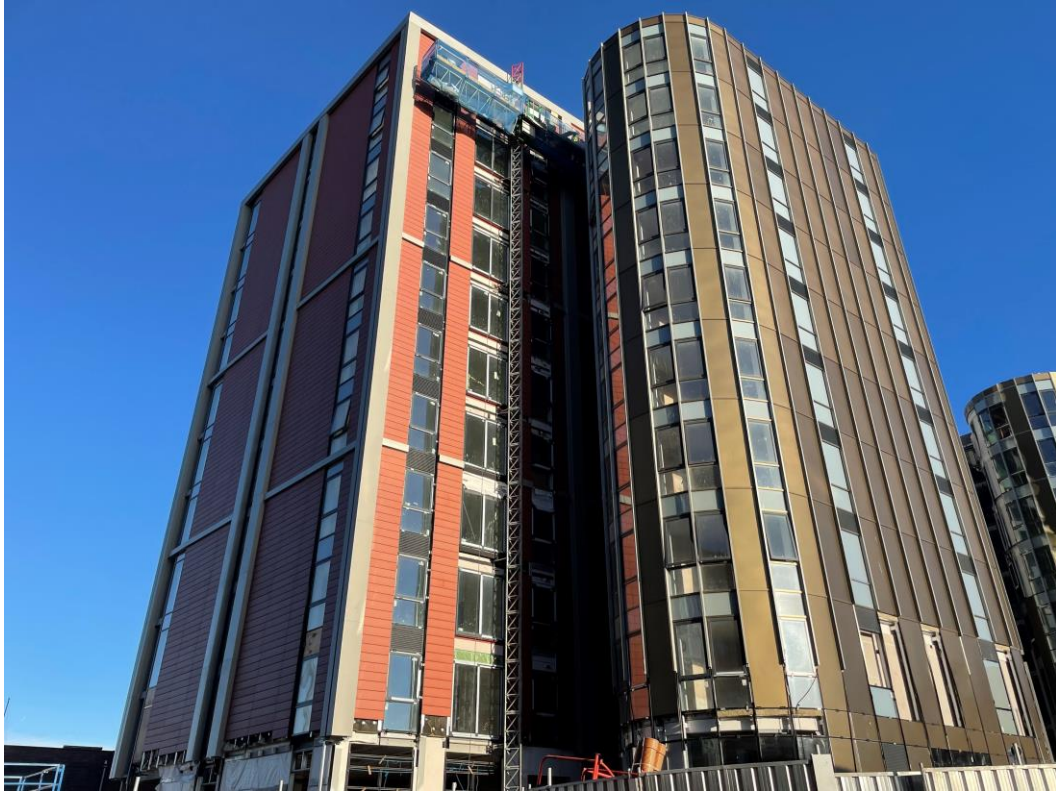
External Cladding remedial works ongoing
