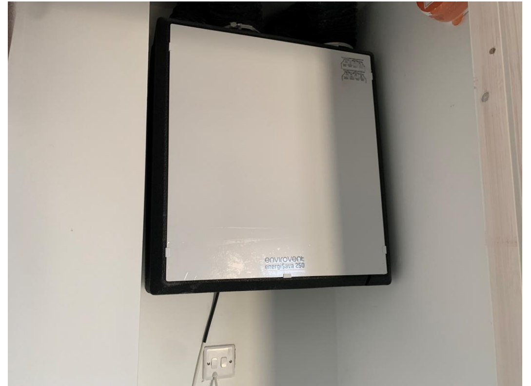
Ventilation system installation ongoing
