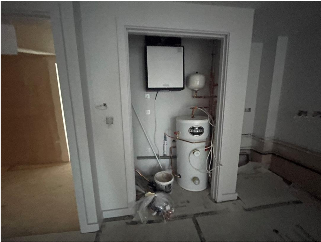
Ventilation system & water cylinder installation ongoing
