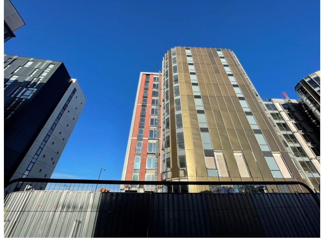
External Cladding remedial works ongoing
