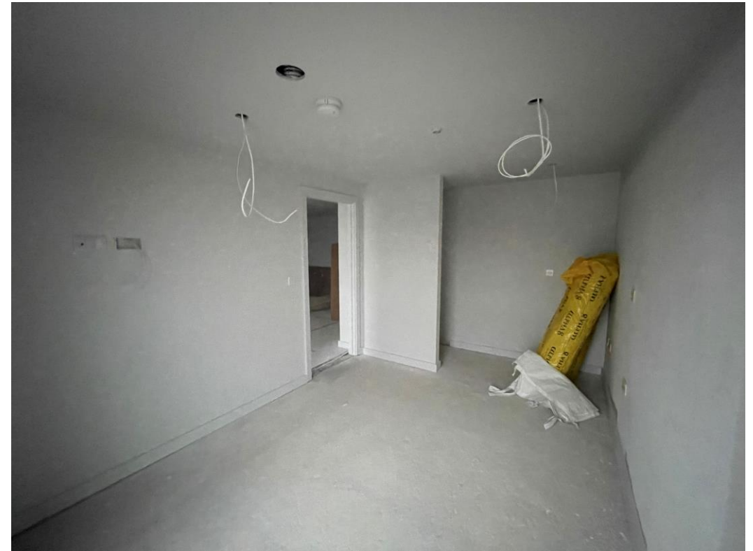
1 st fix electrical installation ongoing
