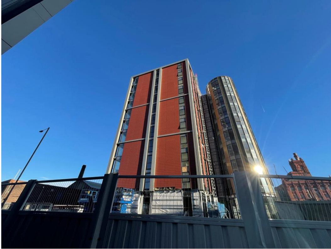
Development viewed from Caryl Street
