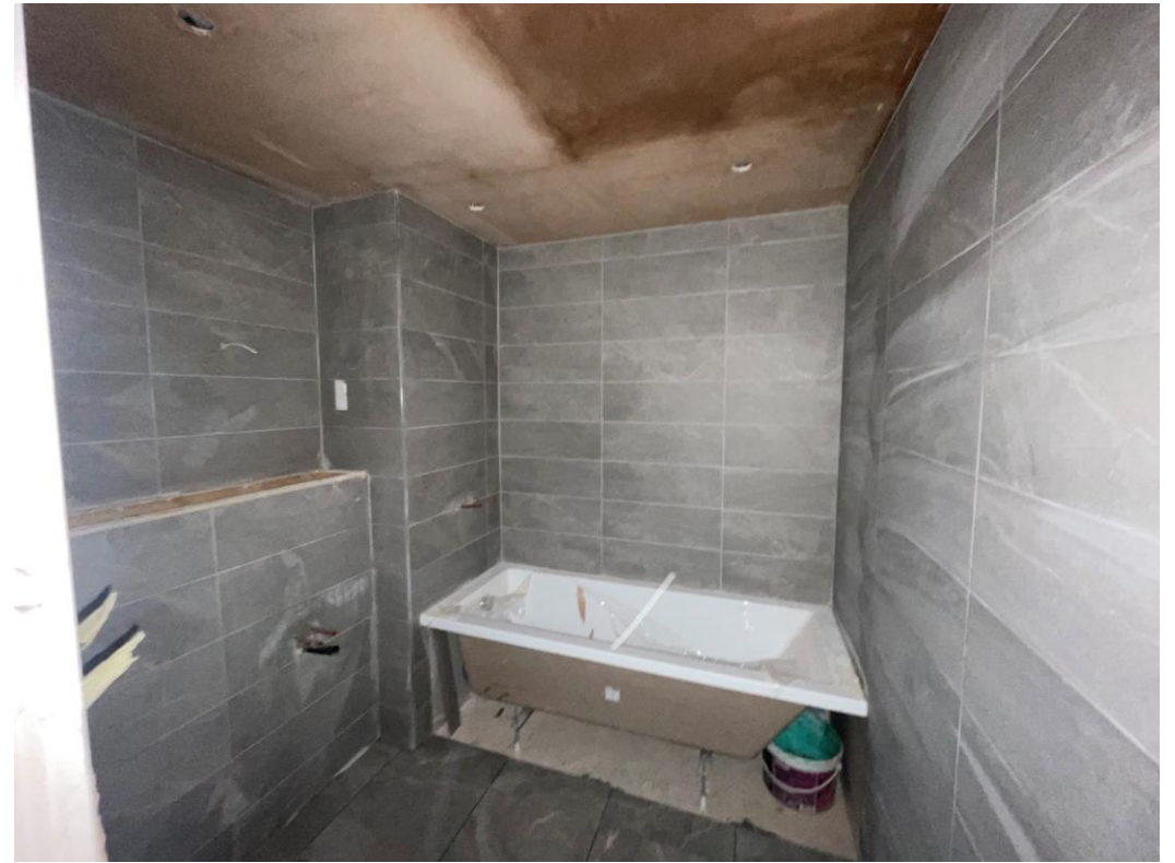
Skim coat applied to bathroom ceiling
