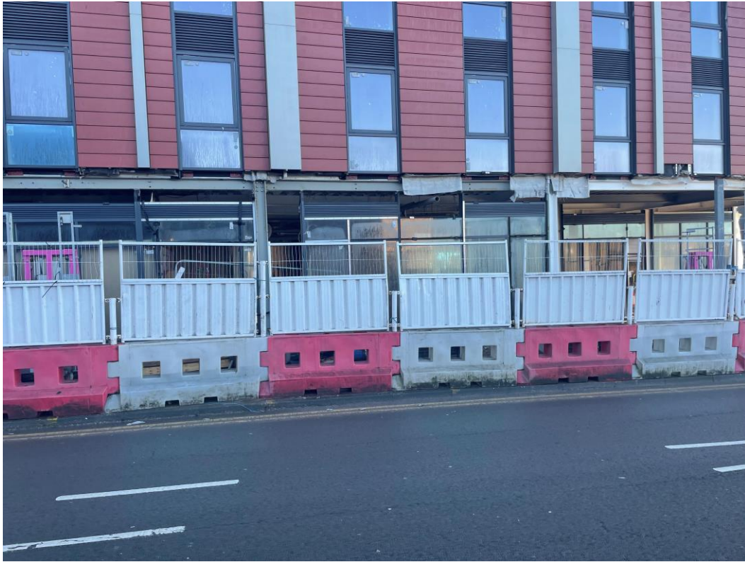
Street hoarding in place on Parliament square
