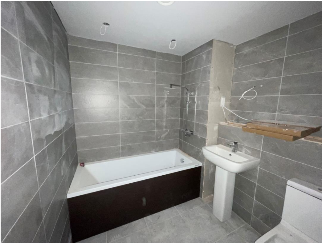
Sanitary & vanity shelf installation ongoing
