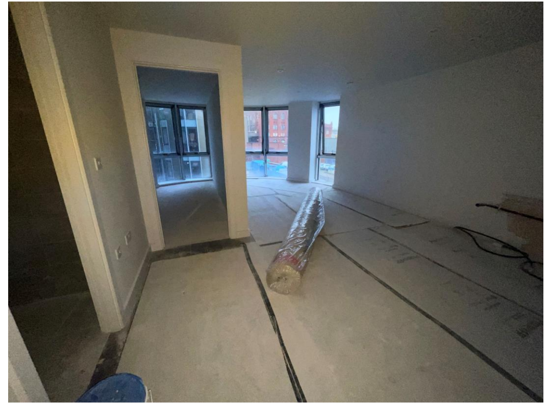
Carpets & underlay on site ready for installation
