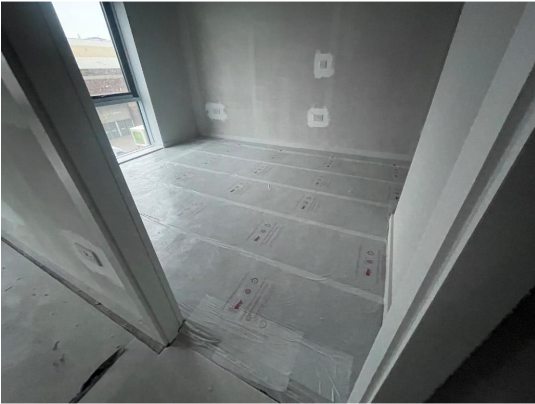
Carpets installation ongoing
