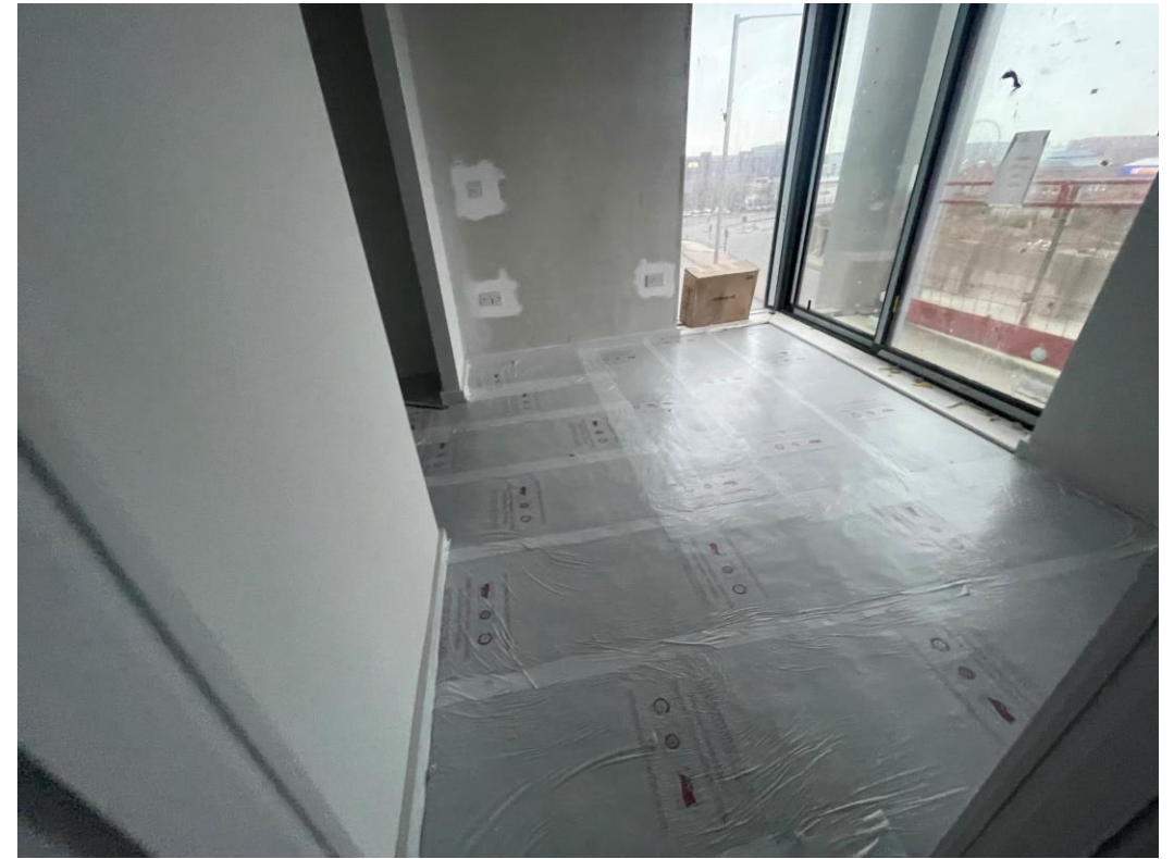
Carpets installation ongoing
