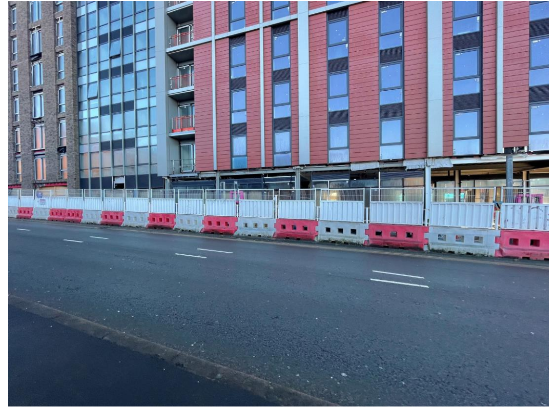
Street hoarding in place on Parliament square
