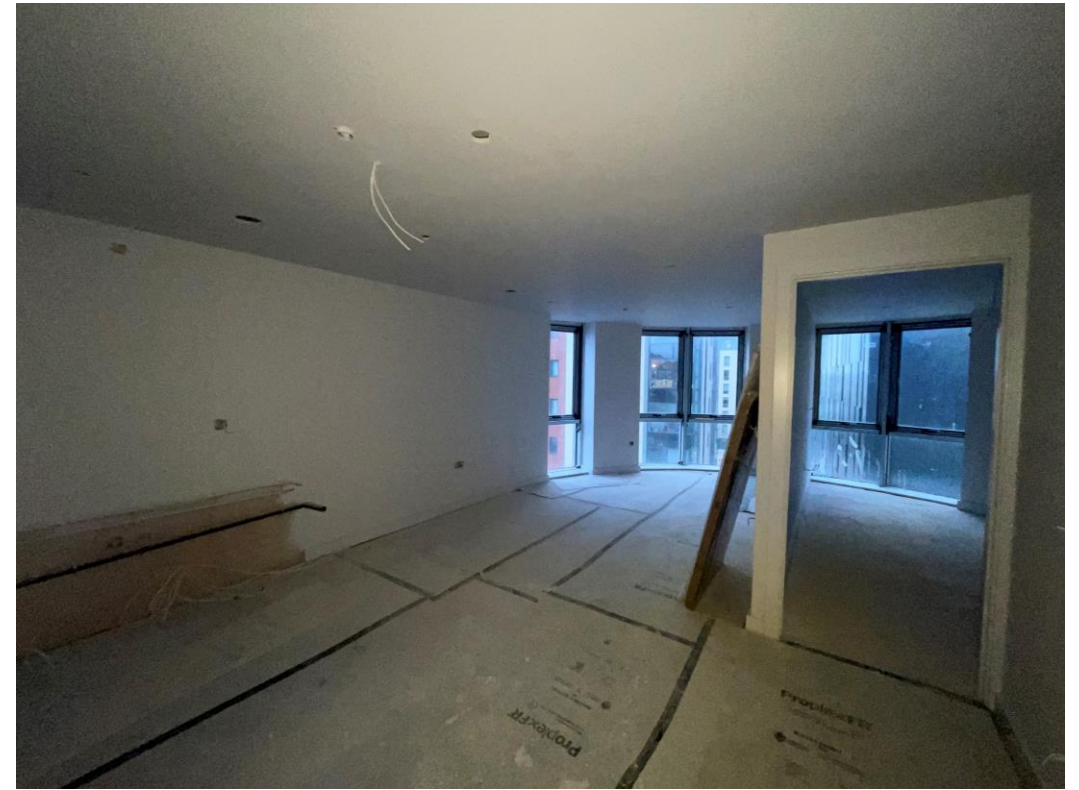
Decoration ongoing to apartments
