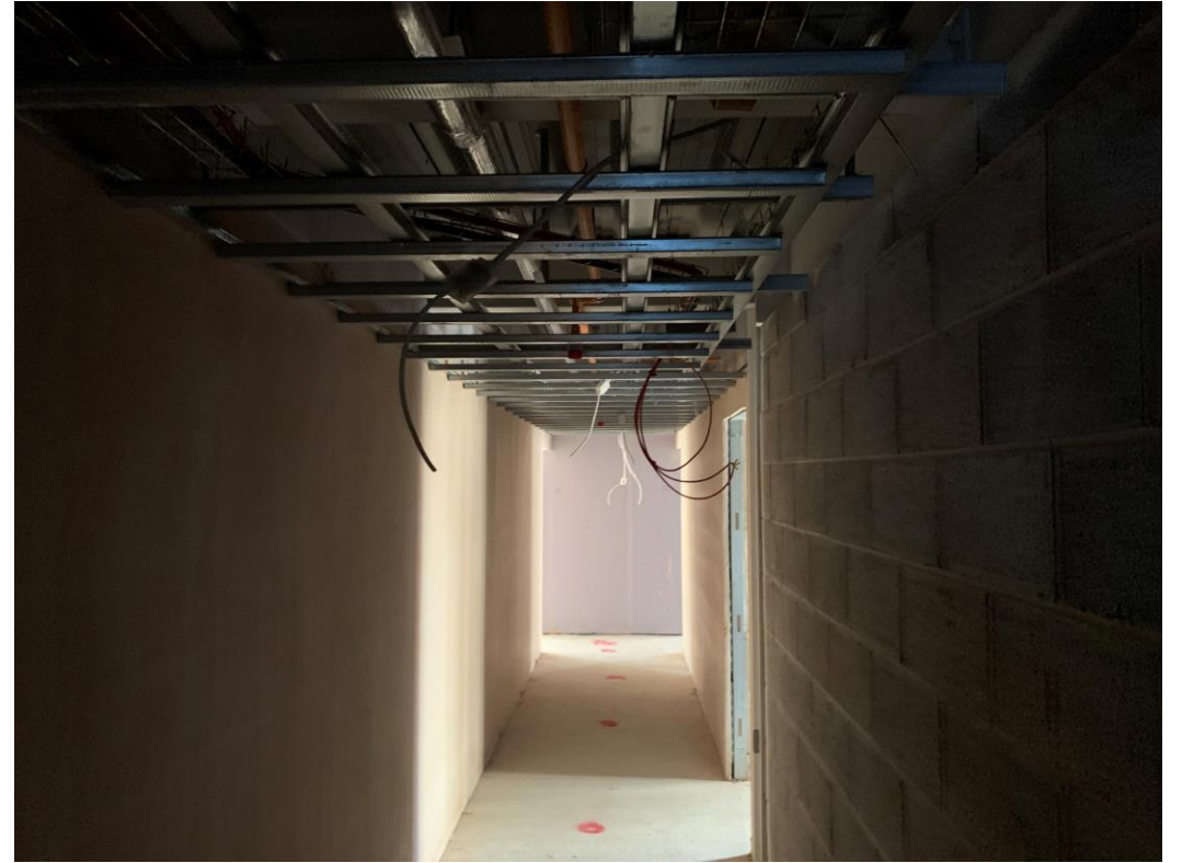
Metal ceiling grid erected to circulation area
