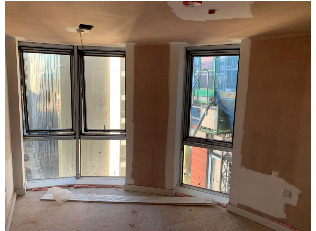
Walls & ceiling skimmed
