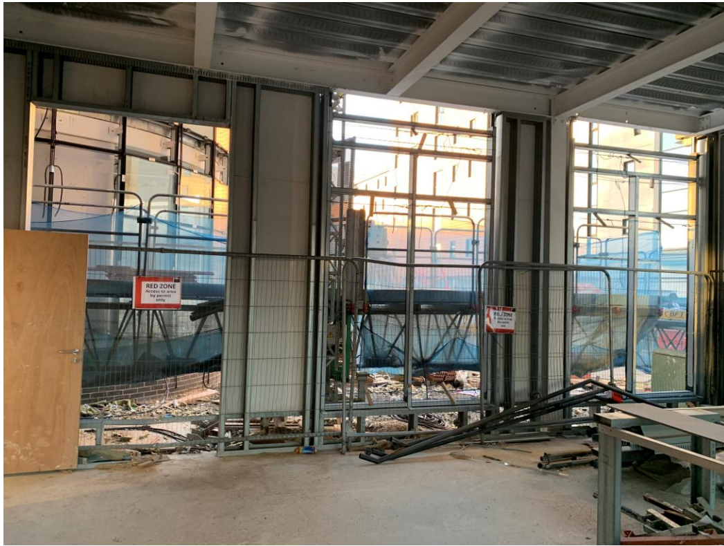
Segregation barriers installed to mass climber areas
