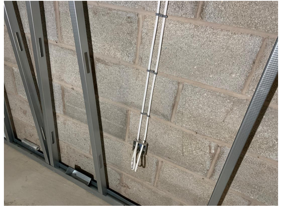
Partitions installed to stair case
