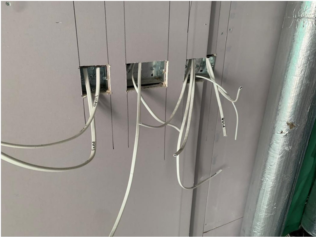
1 st fix electrics for sockets
