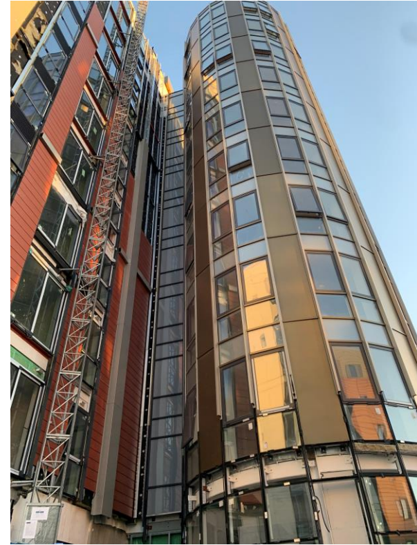
External cladding remedial works and reinstated
