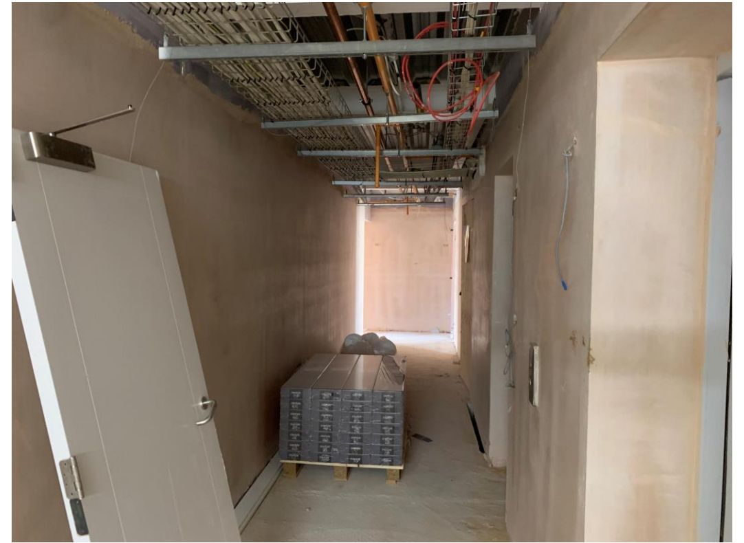
Ceiling grid erected to circulation area
