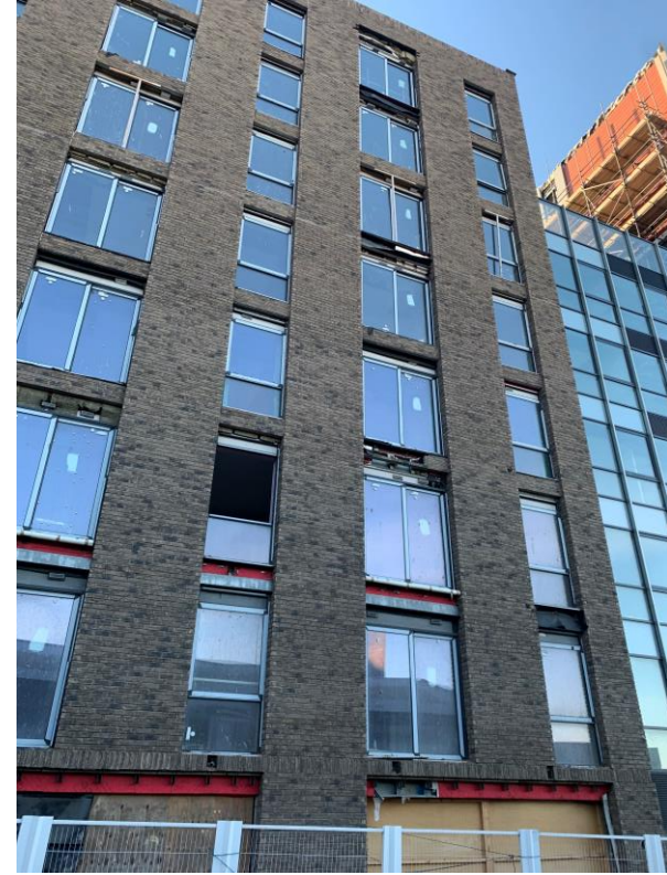
Development viewed from Parliament Street. External works ongoing
