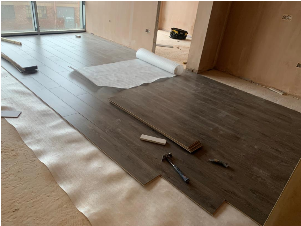
Laminate floor installation
