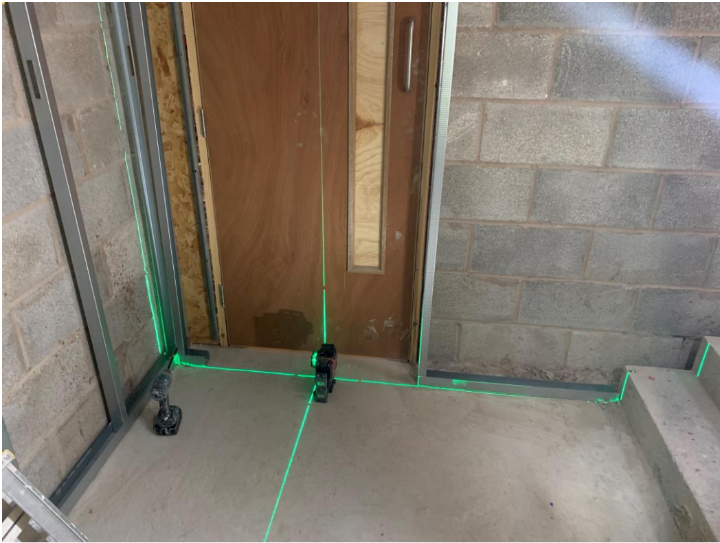
Partitions installed to stair case
