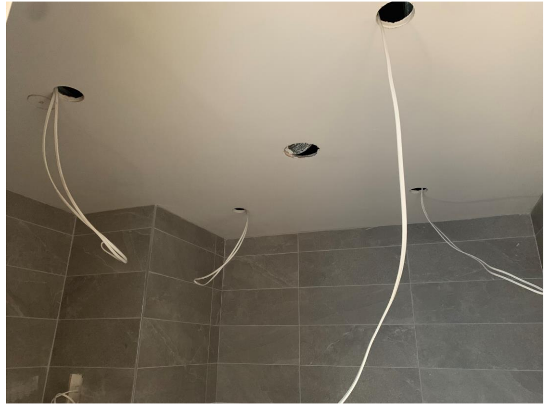
1 st fix electrics for spotlight
