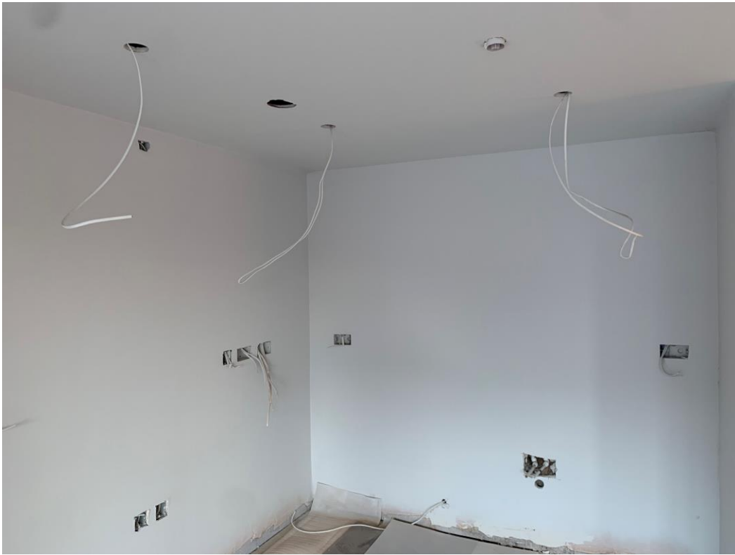
1 st coat decoration to kitchen. 1 st fix electrics ongoing
