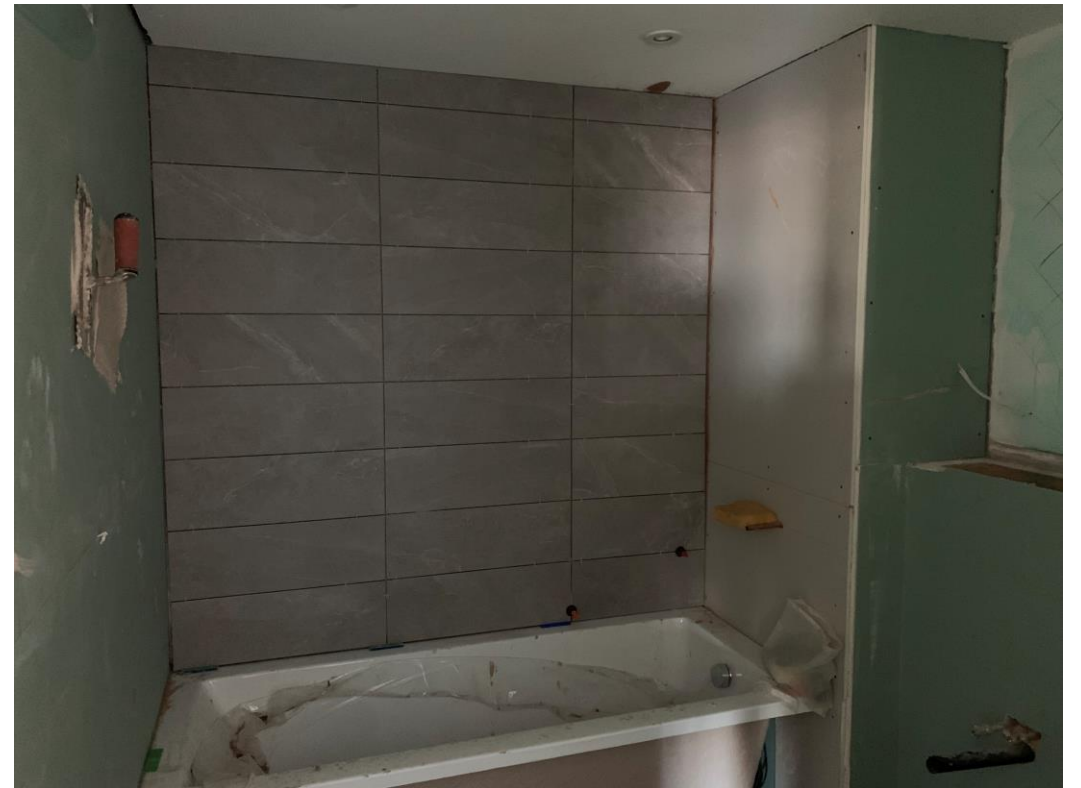
Bath installed. Tiling has commenced
