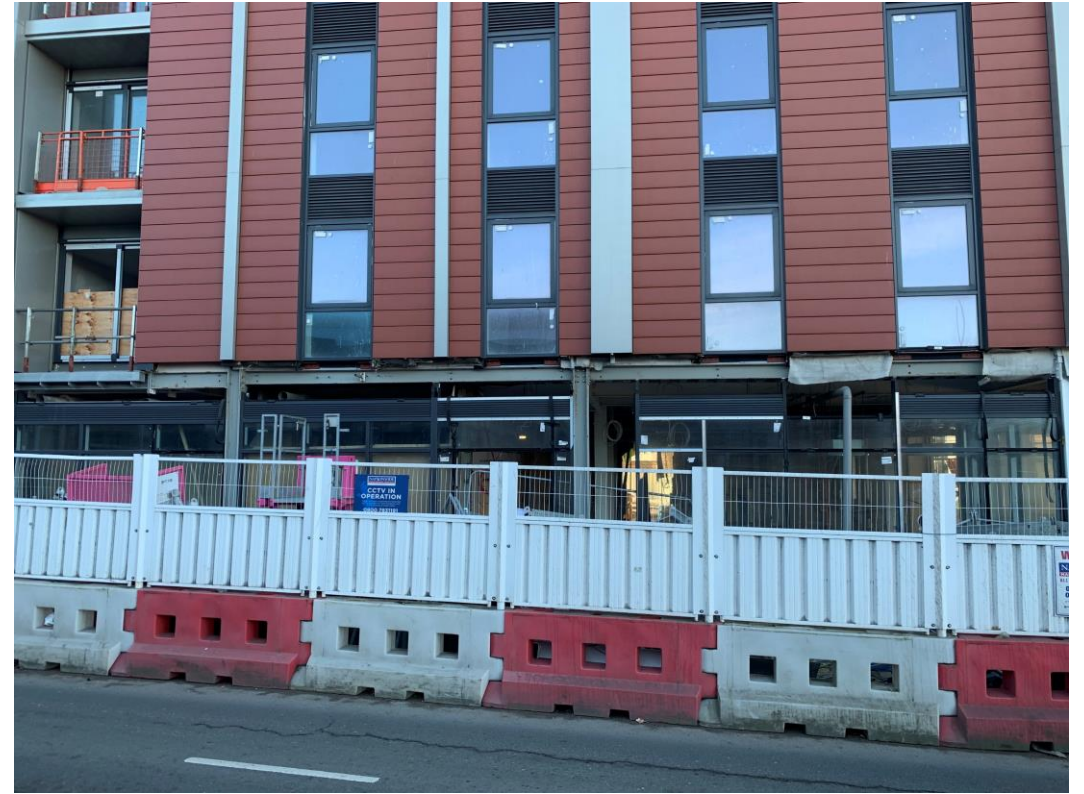
Site hoarding adjusted to facilitate curtain wall installation
