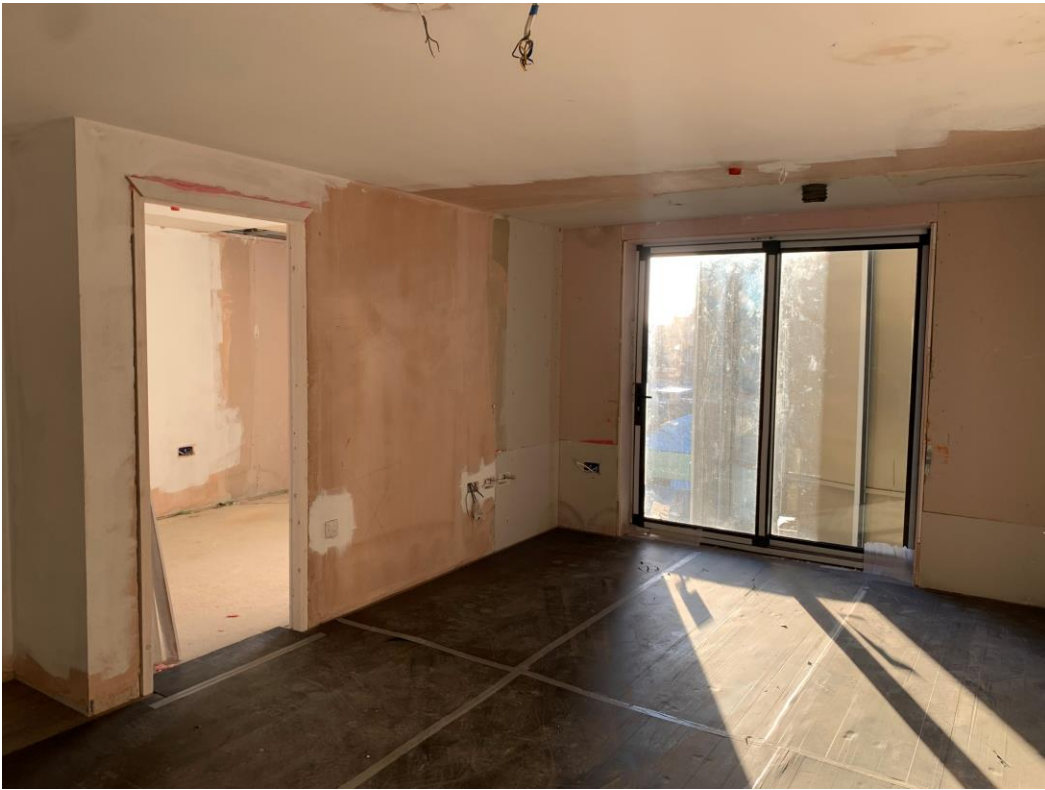
Flooring finishes installed & protected
