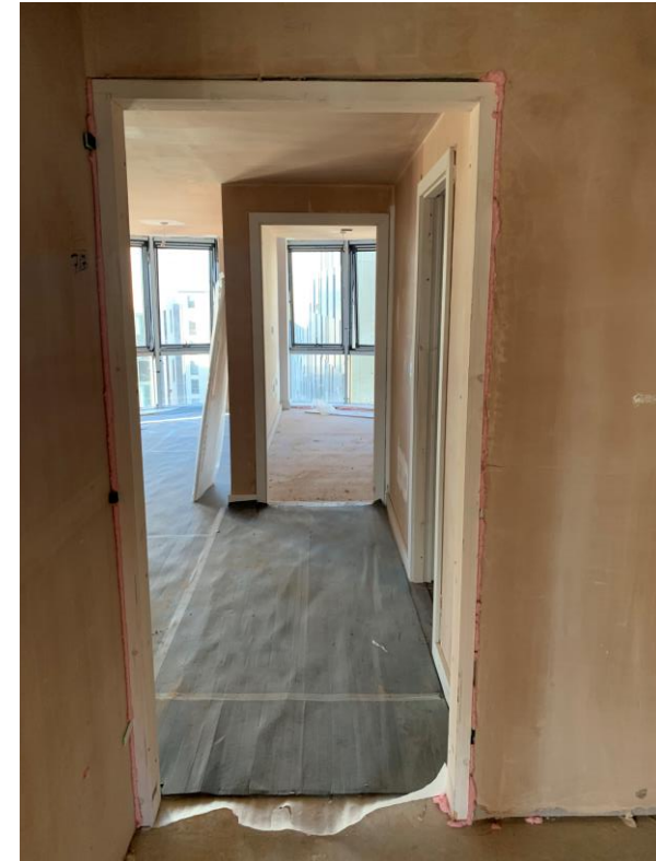
Door frames and architraves installed
