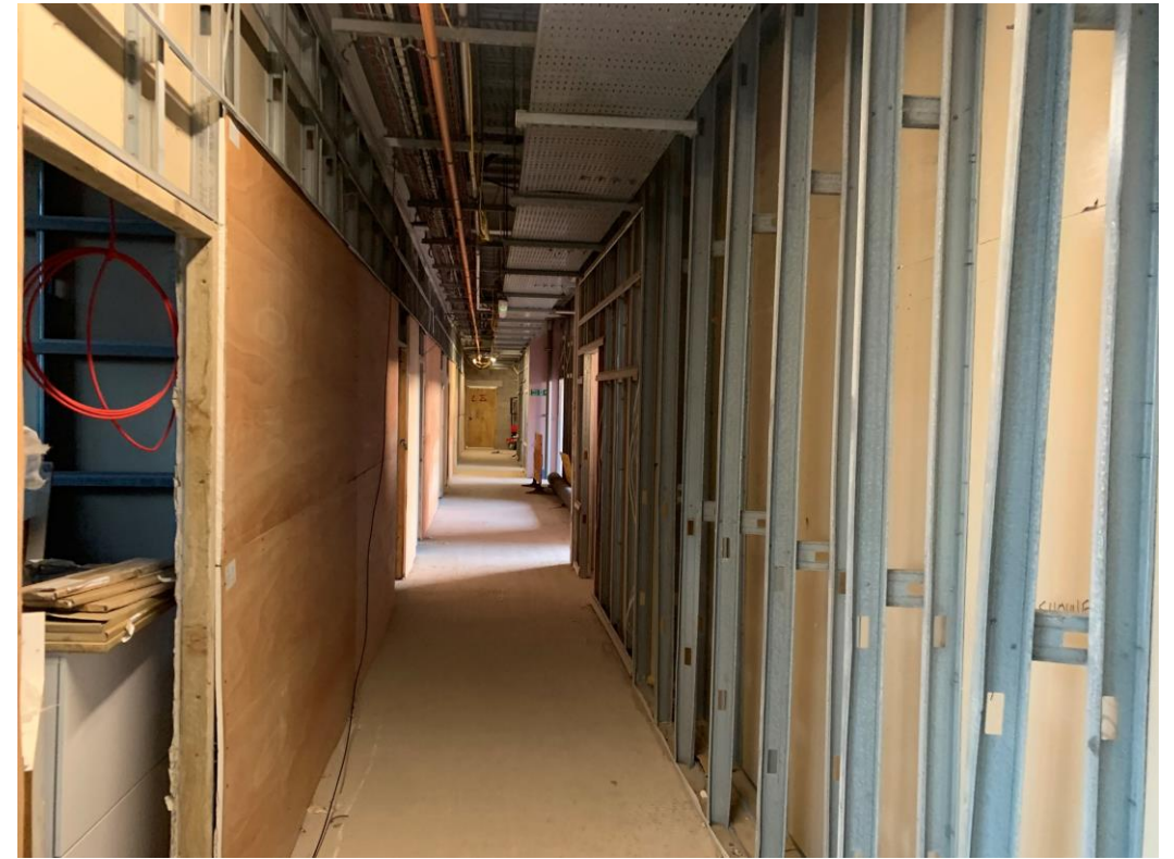
Partitions installation to circulation area complete
