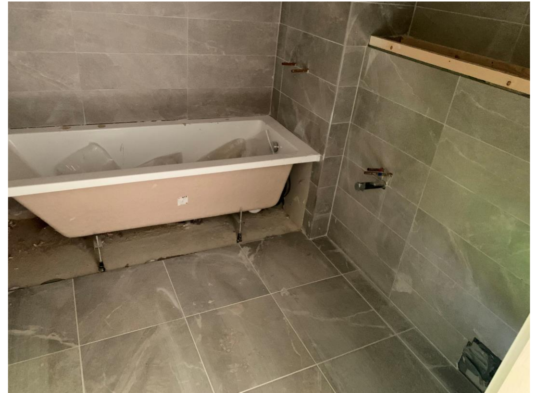
Bath installed. Floor & wall tiling complete
