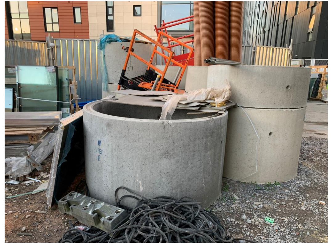
Concrete manhole rings
