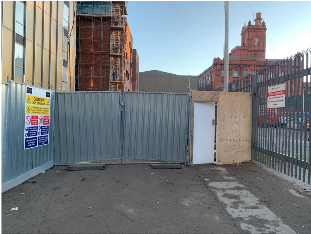
New Secure site entrance
