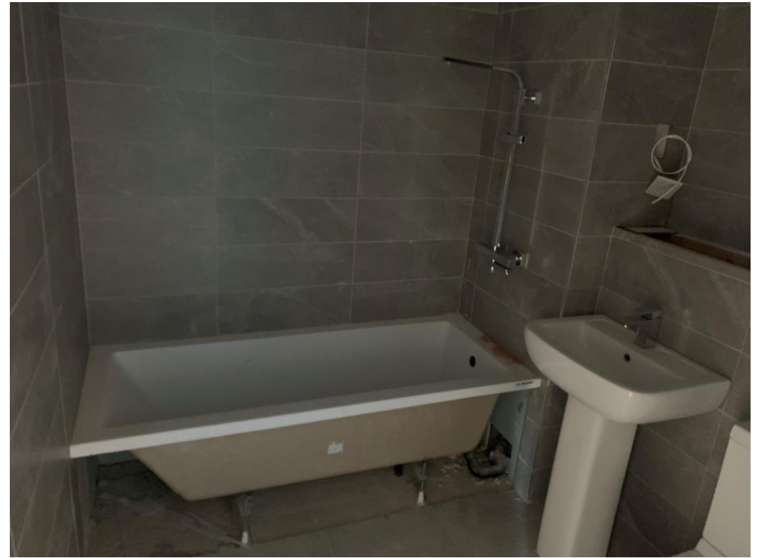
Bath, shower & WHB. Floor & wall tiling complete
