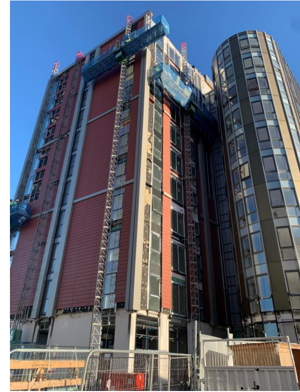
External cladding remedial works and reinstated
