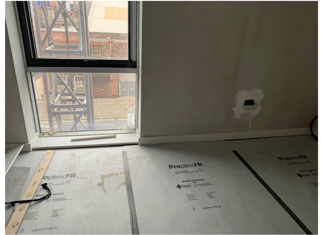
Architraves & window bored installed. Floor finishes installed & protected
