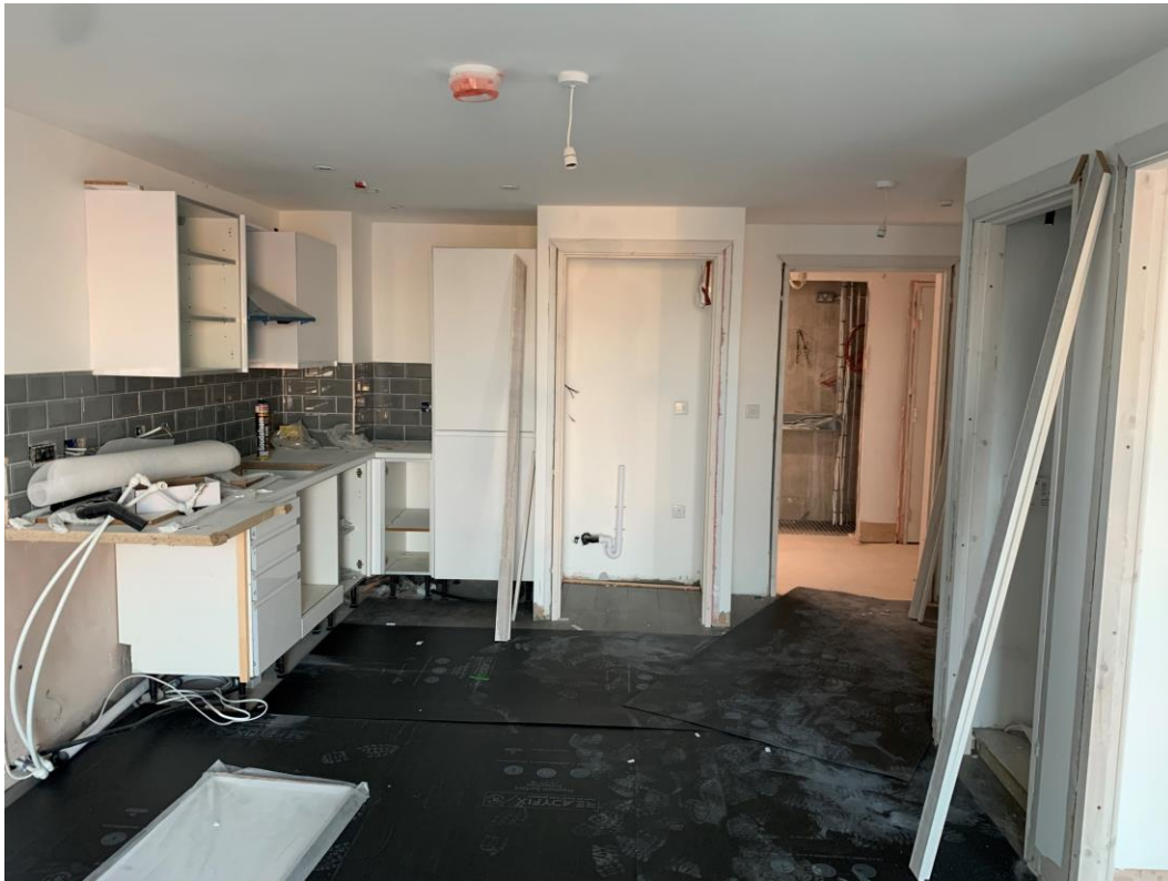
Removal of kitchen. Floor finishes installed & protected
