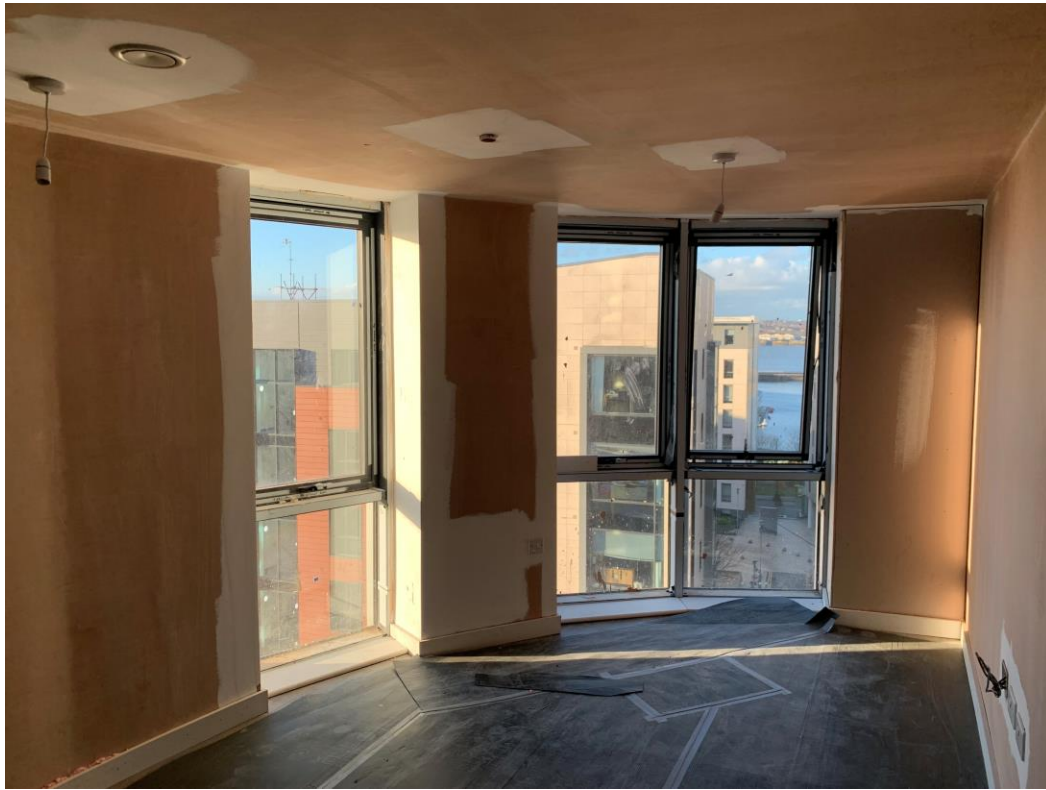
Walls & ceiling skimmed. Floor finishes installed & protected
