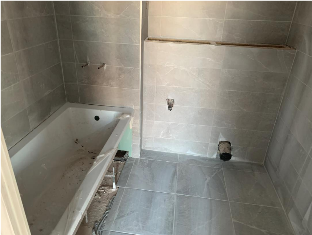
Bath installed. Floor & wall tiling complete
