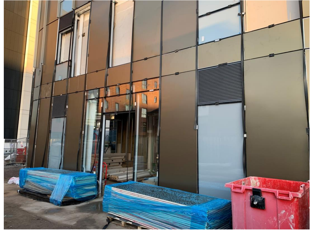
External cladding remedial works and reinstated
