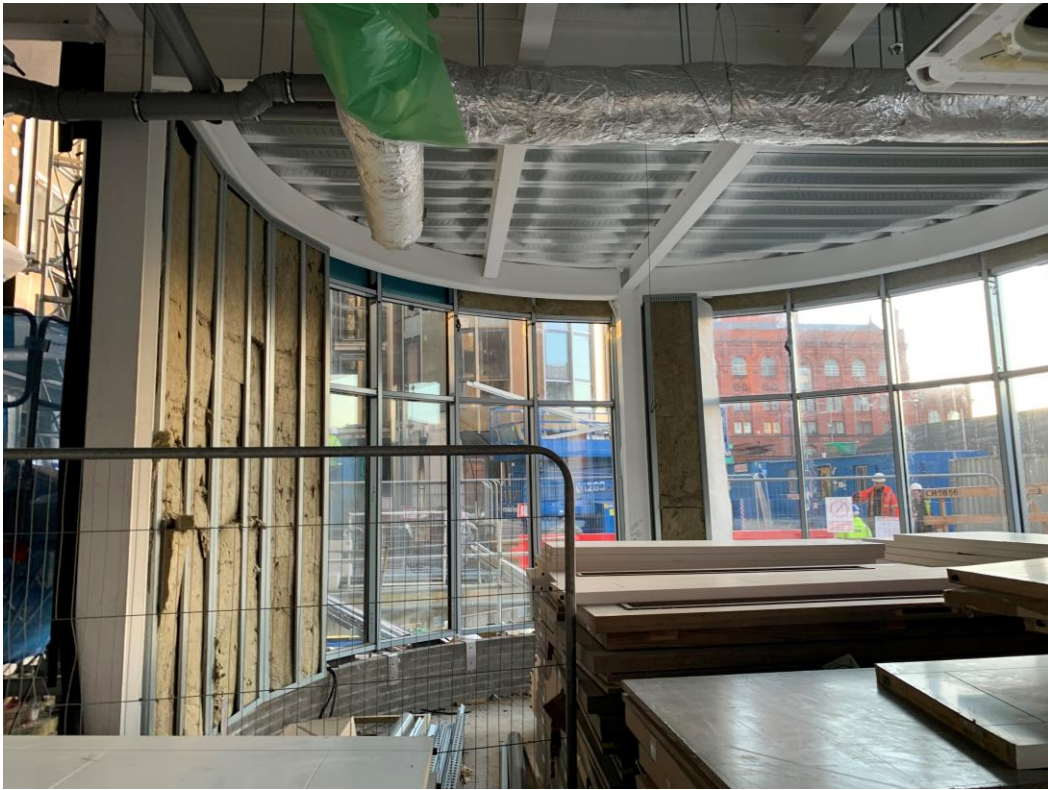
Removal of old doors ongoing
