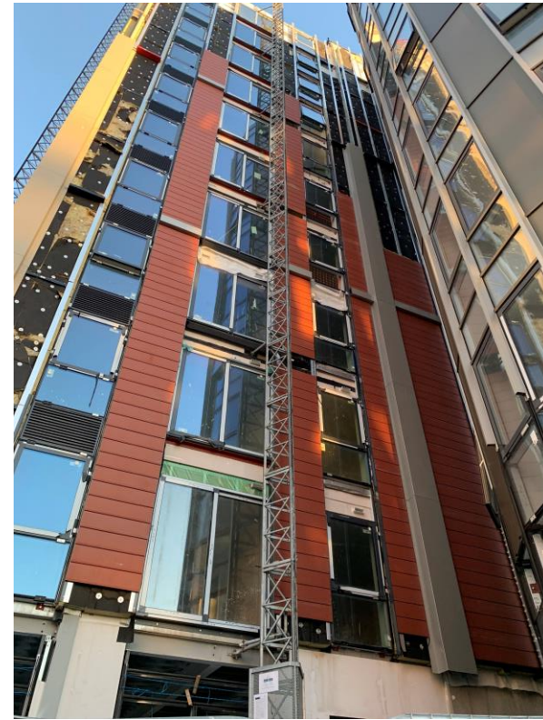
External cladding remedial works and reinstated
