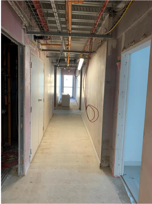
Boarding to circulation areas ongoing
