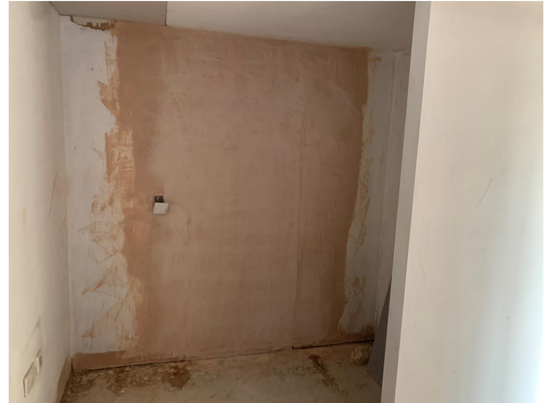
Jack & Jill bathroom door blocked up, boarded & skimmed
