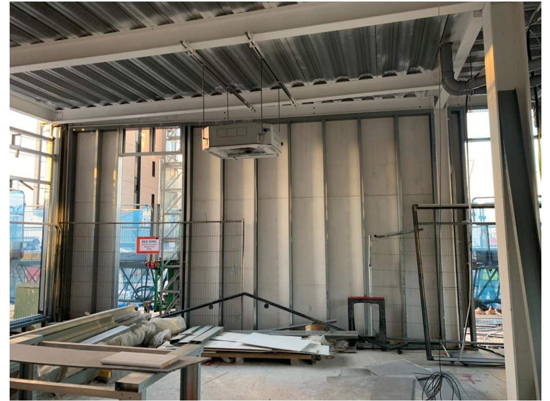
Segregation barriers installed to mass climber areas
