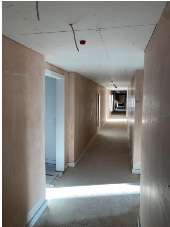
Ceilings boarded and walls skimmed to circulation areas
