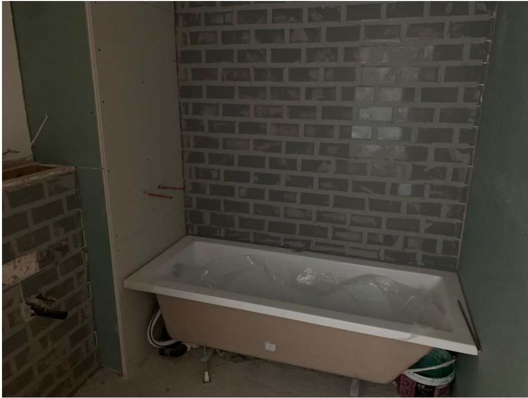
Bath installed. Ready for tiling
