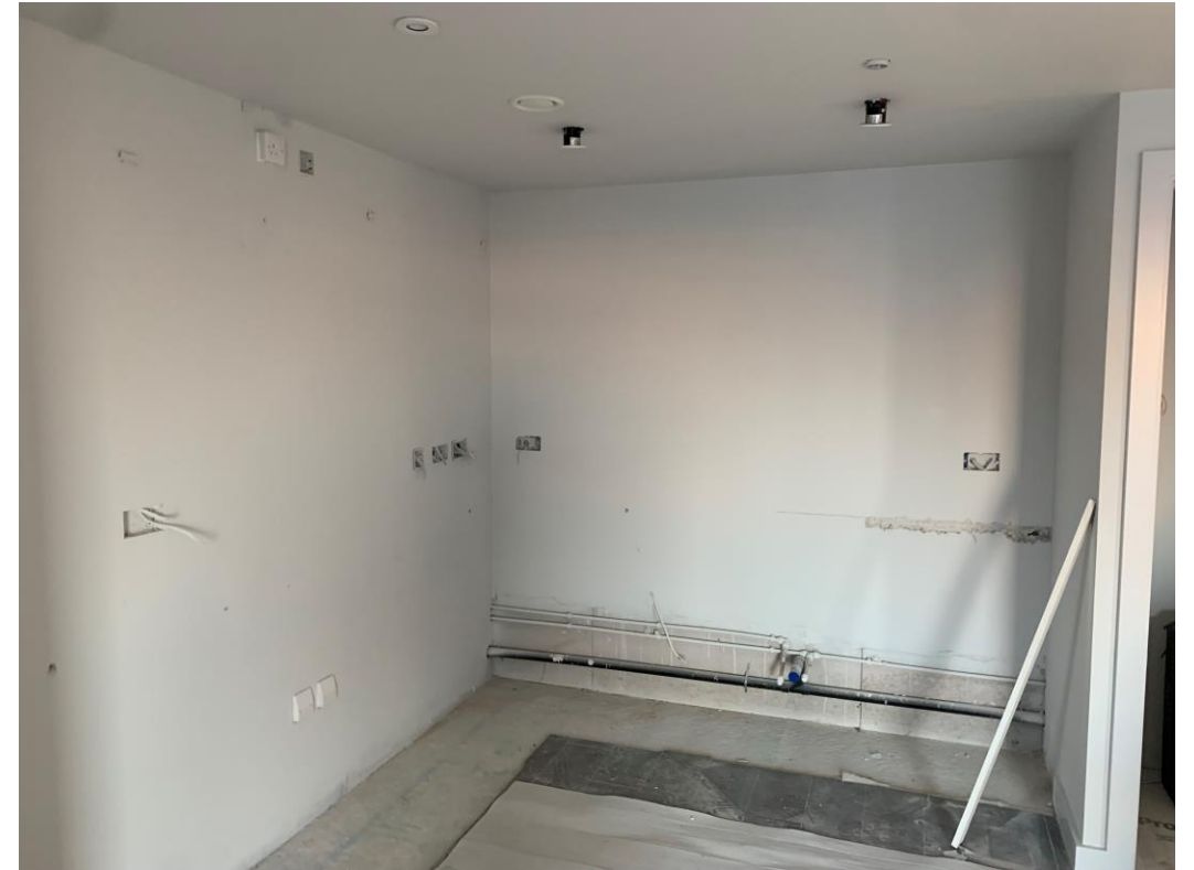
1 st coat decoration to kitchen area
