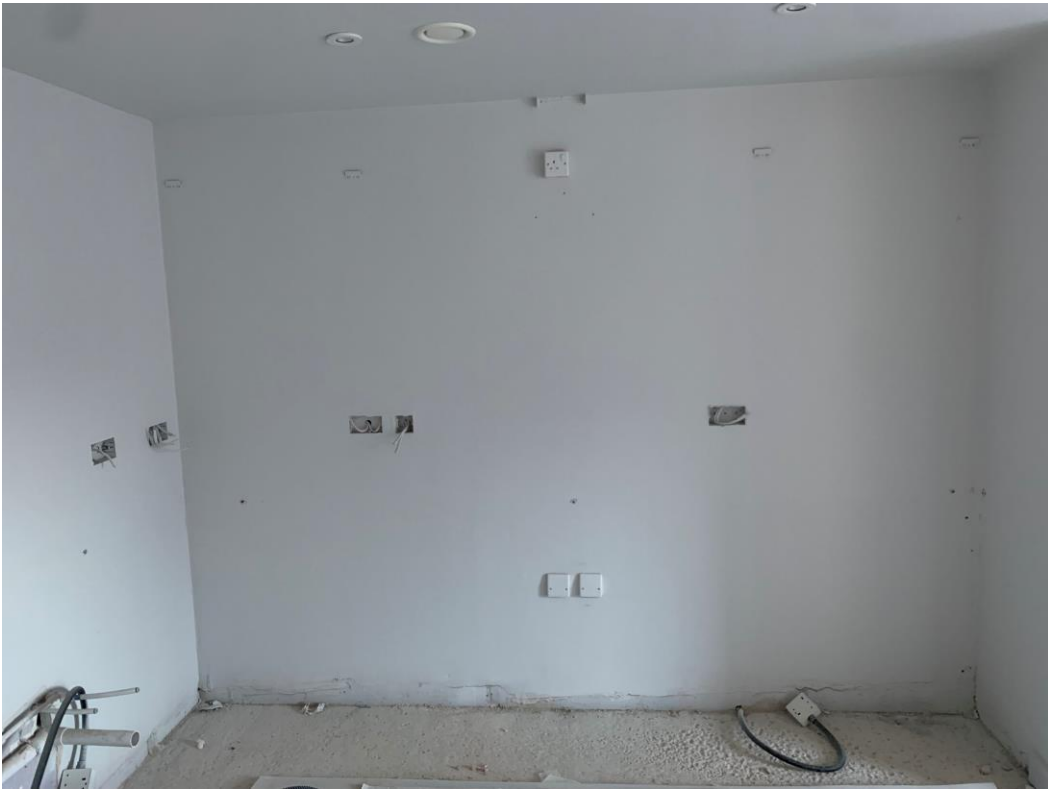
1 st coat decoration to kitchen area
