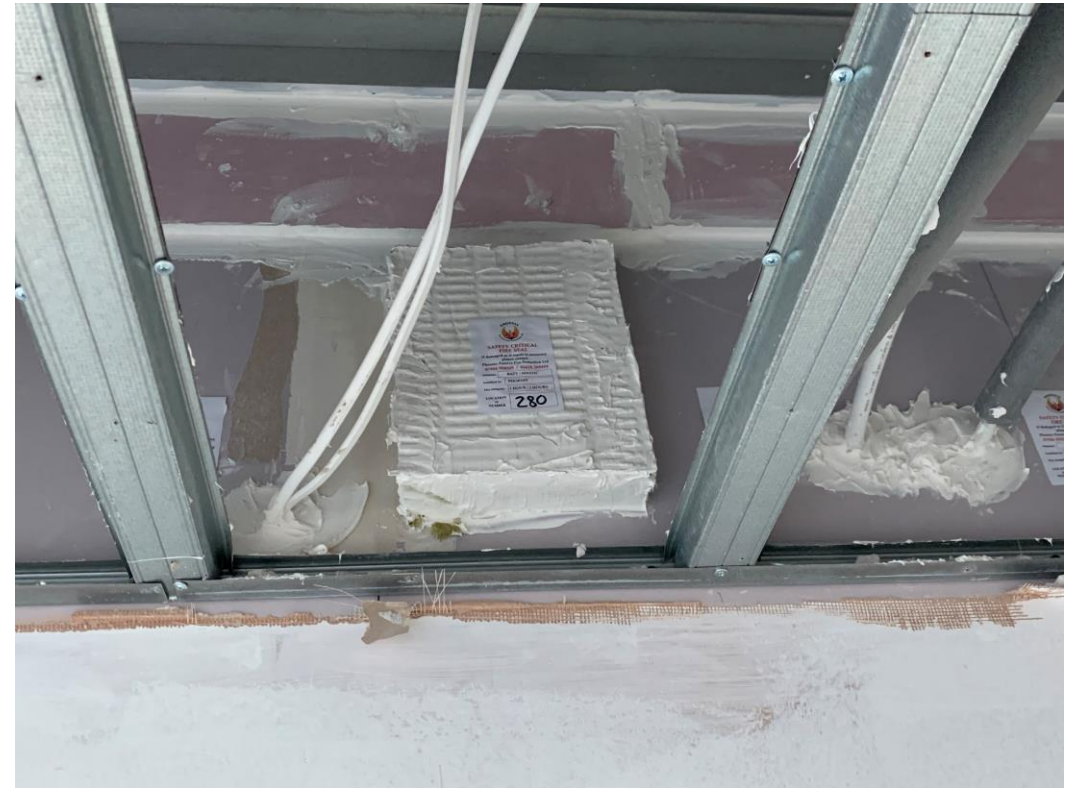
Fire stopping to apartment areas
