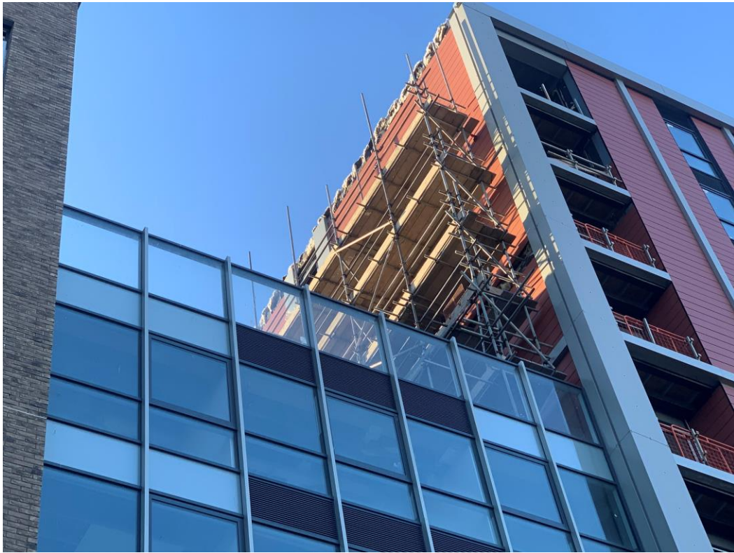
Scaffolding erected to terrace elevation. Cladding installation has commenced
