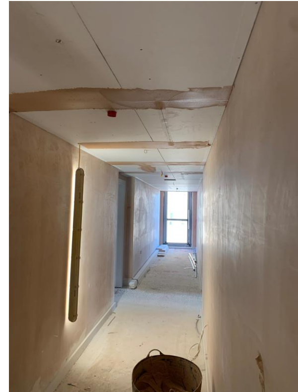
Ceilings boarded and walls skimmed to circulation areas
