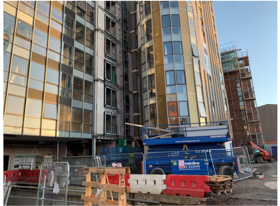
External cladding remedial works and reinstated
