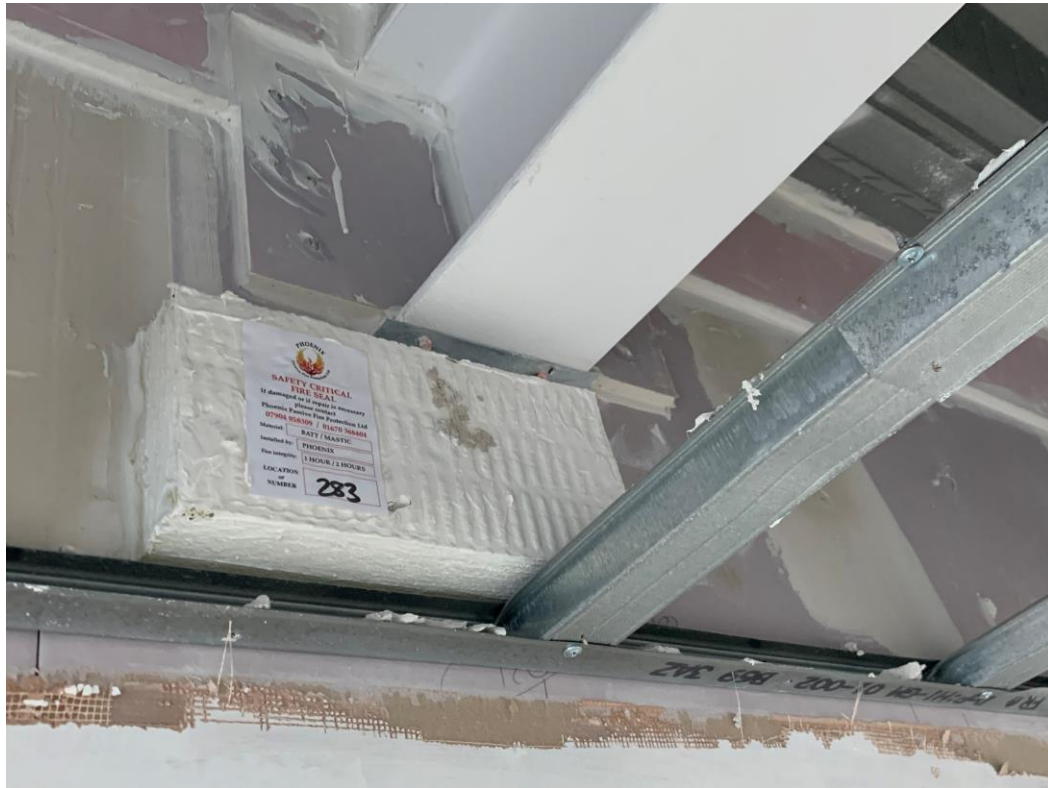
Fire stopping to apartment areas
