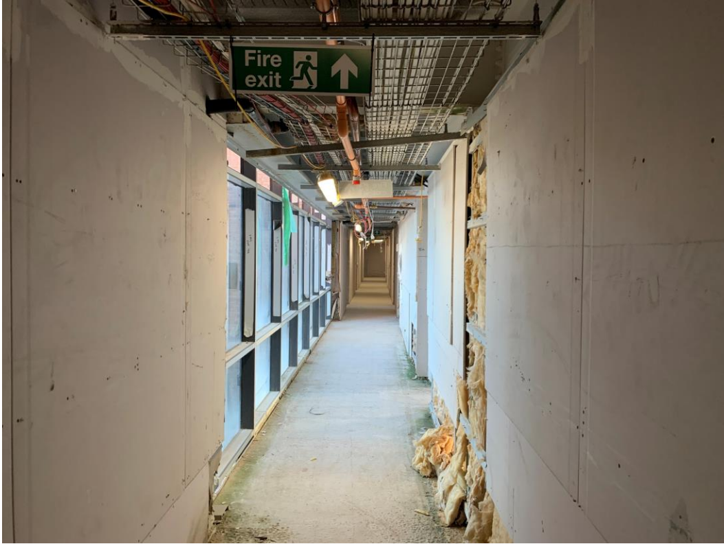
Insulation & boarding of circulation areas ongoing
