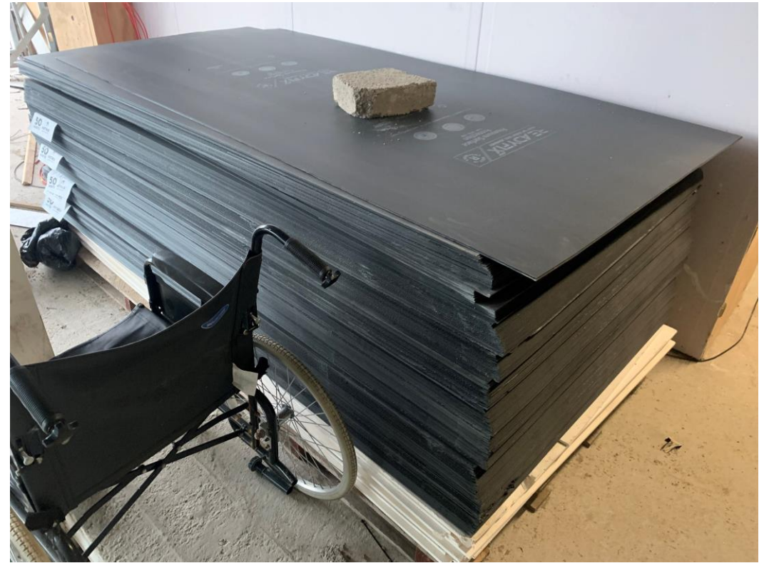
Corex sheets onsite for floor protection
