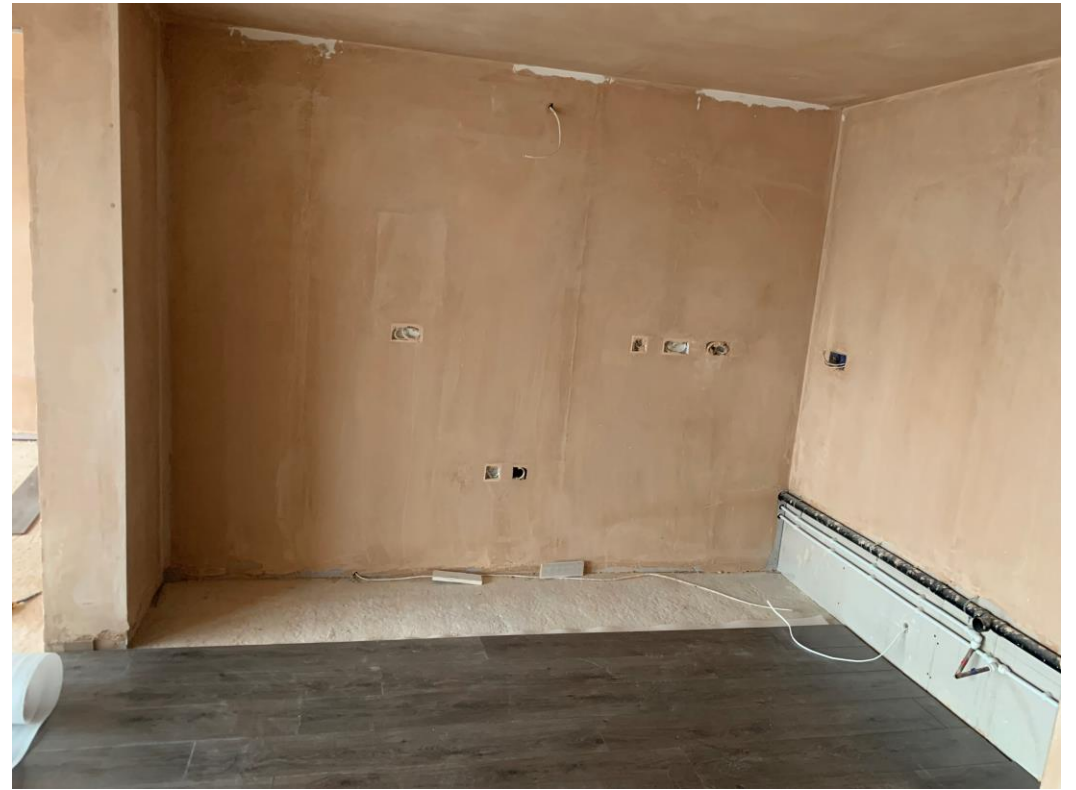
Laminate floor installation
