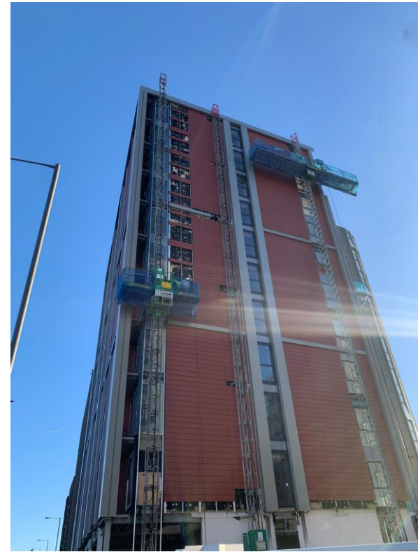
External cladding remedial works and reinstated
