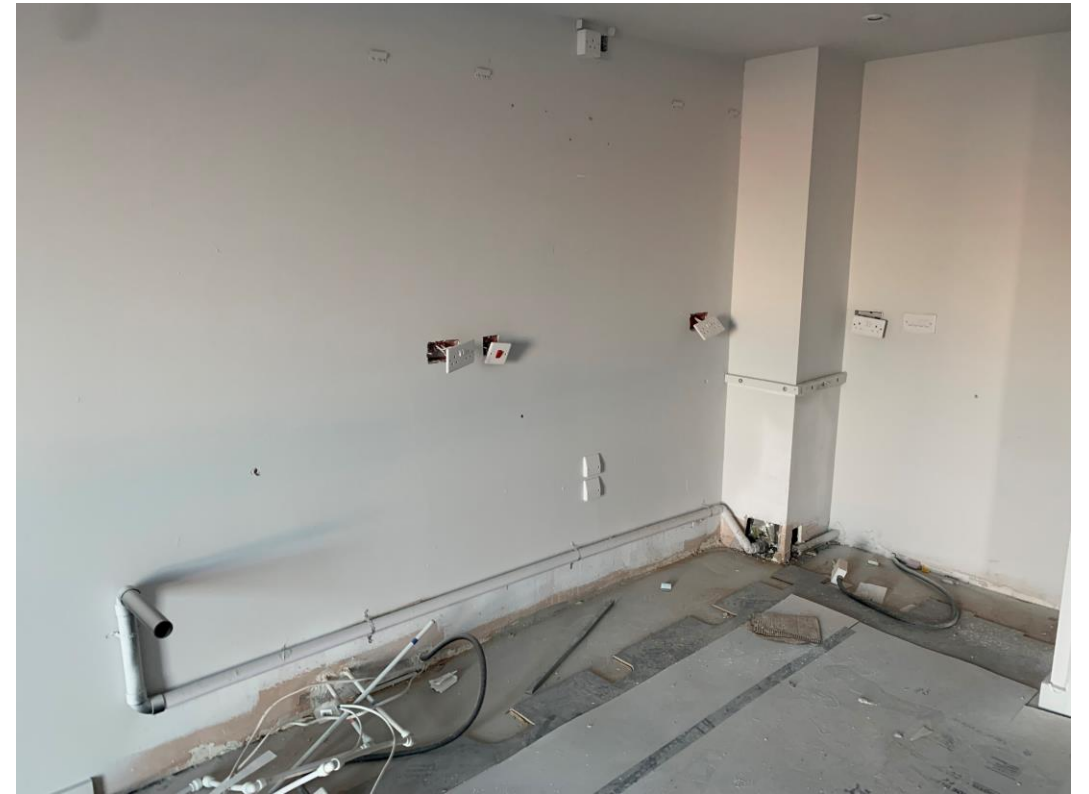
Ceilings and walls 1 st decoration coat. 2 nd fix electrics ongoing
