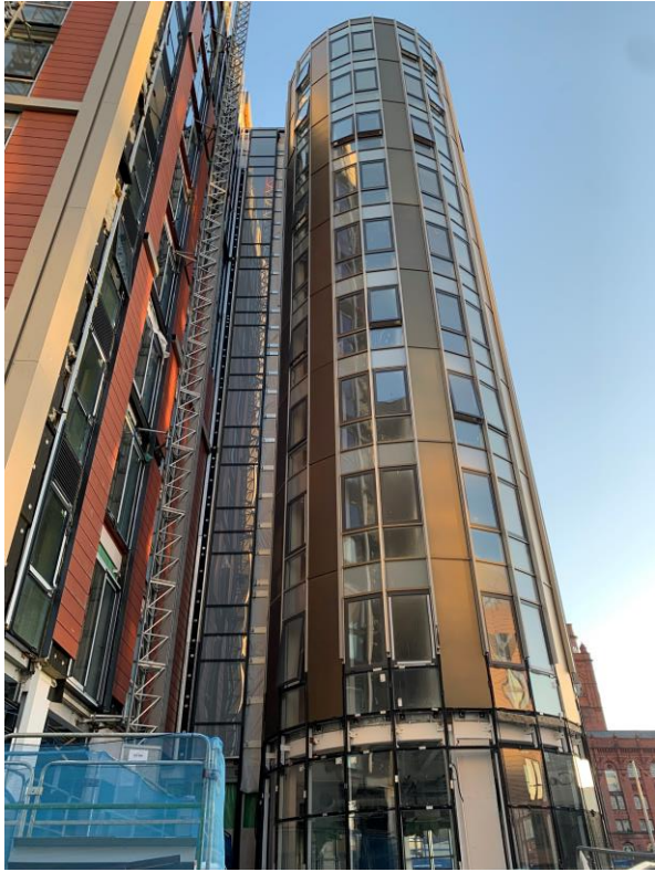
External cladding remedial works and reinstated
