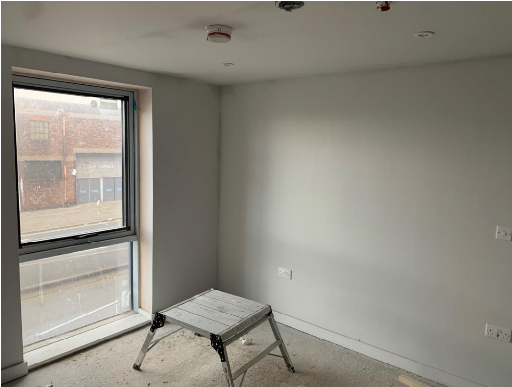
Ceilings and walls 1 st decoration coat
