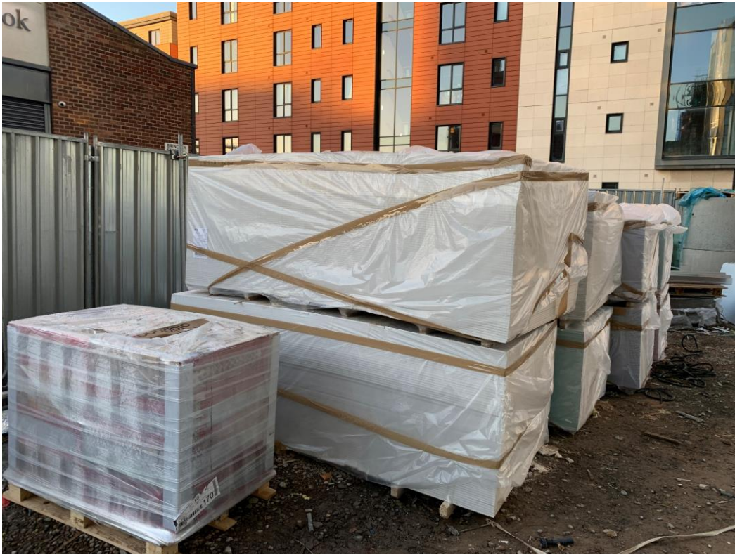
Plasterboard & tiling material
