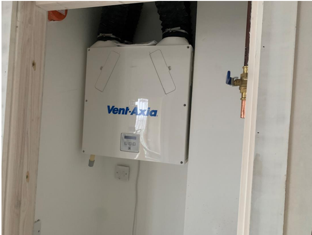
Old heating ventilation
