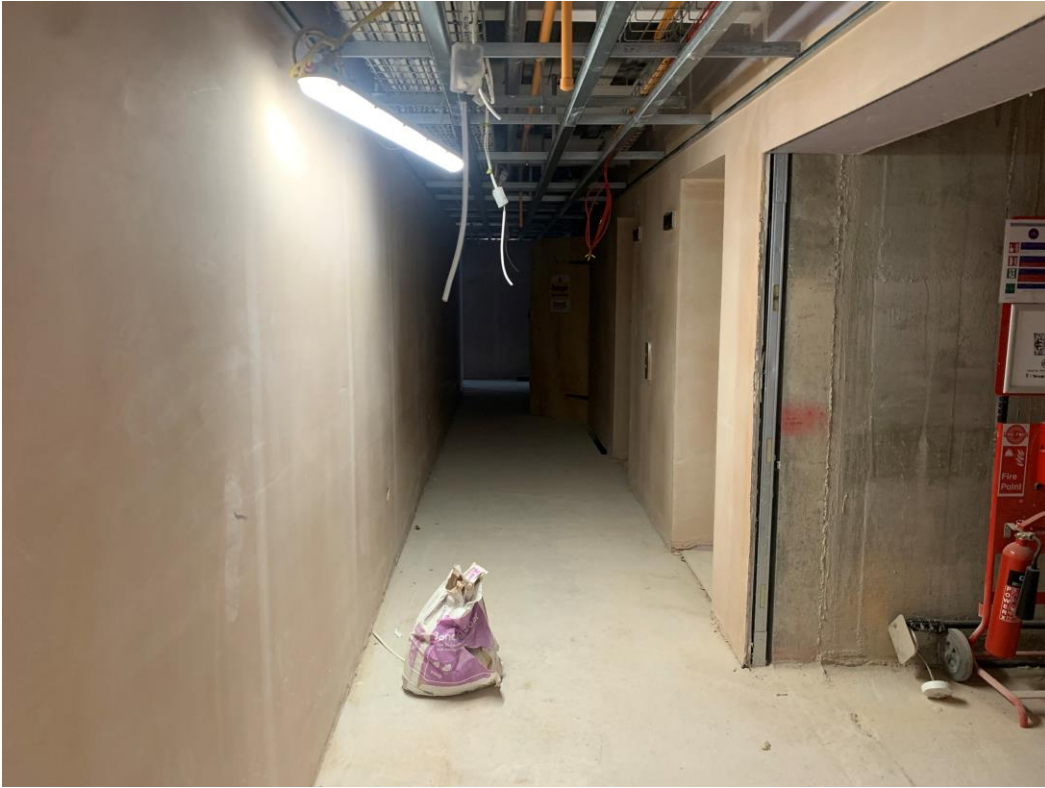
Celling grid installed to lift area
