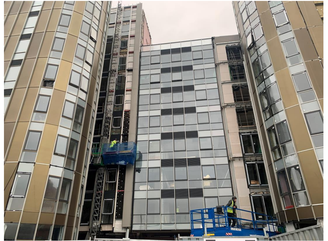
External cladding remedial works and reinstated
