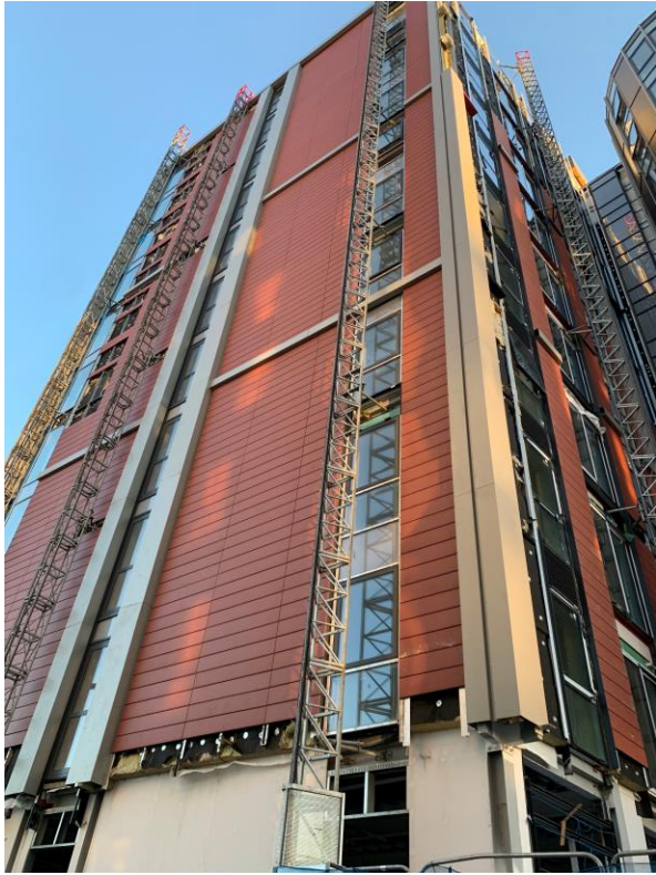
External cladding remedial works and reinstated
