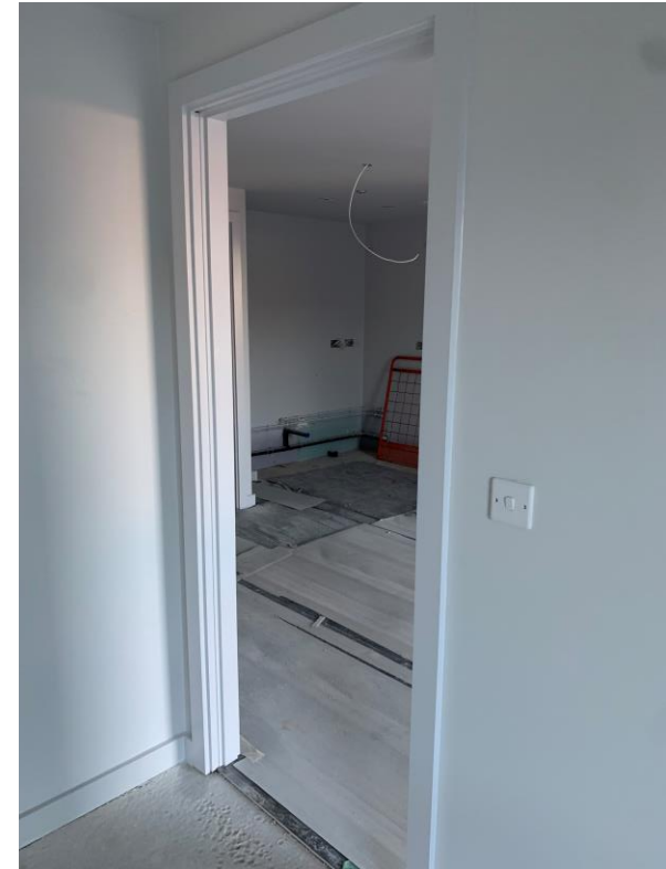
Door Linings, skirting board & architrave installed
