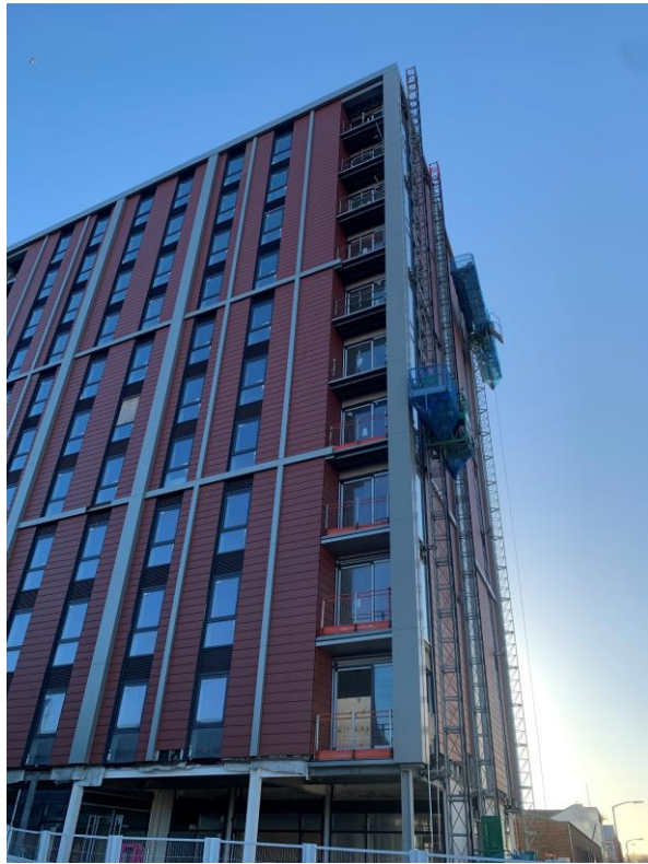
Development viewed from Parliament Street. External works ongoing
