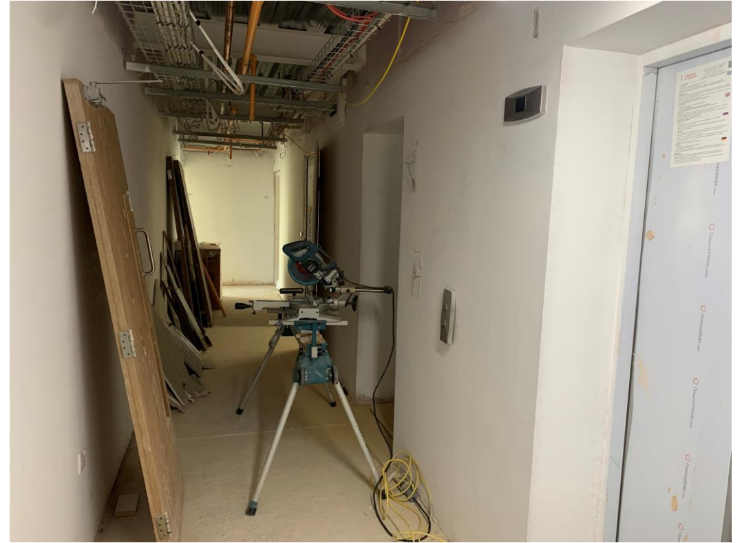
Lift area works ongoing
