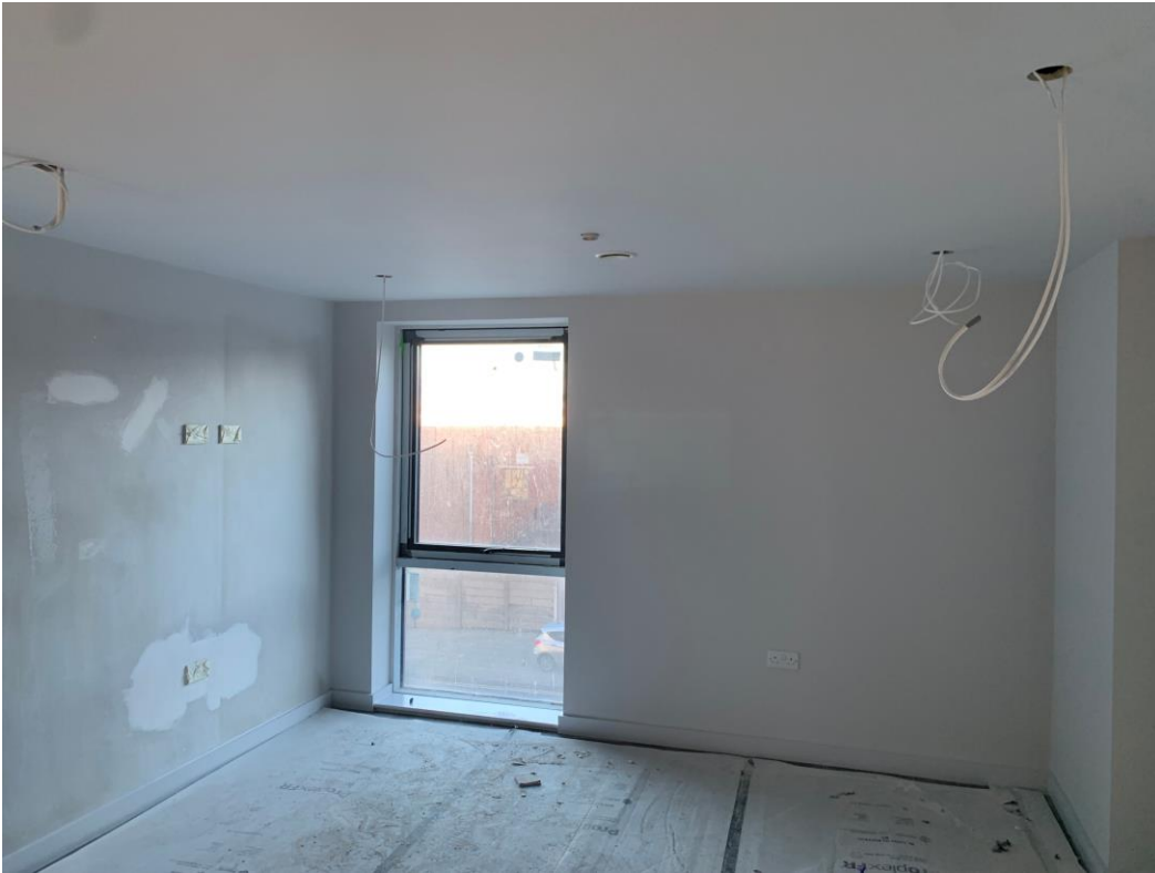
Skirting boards, window boards installed. Floors finishes installed & protected
