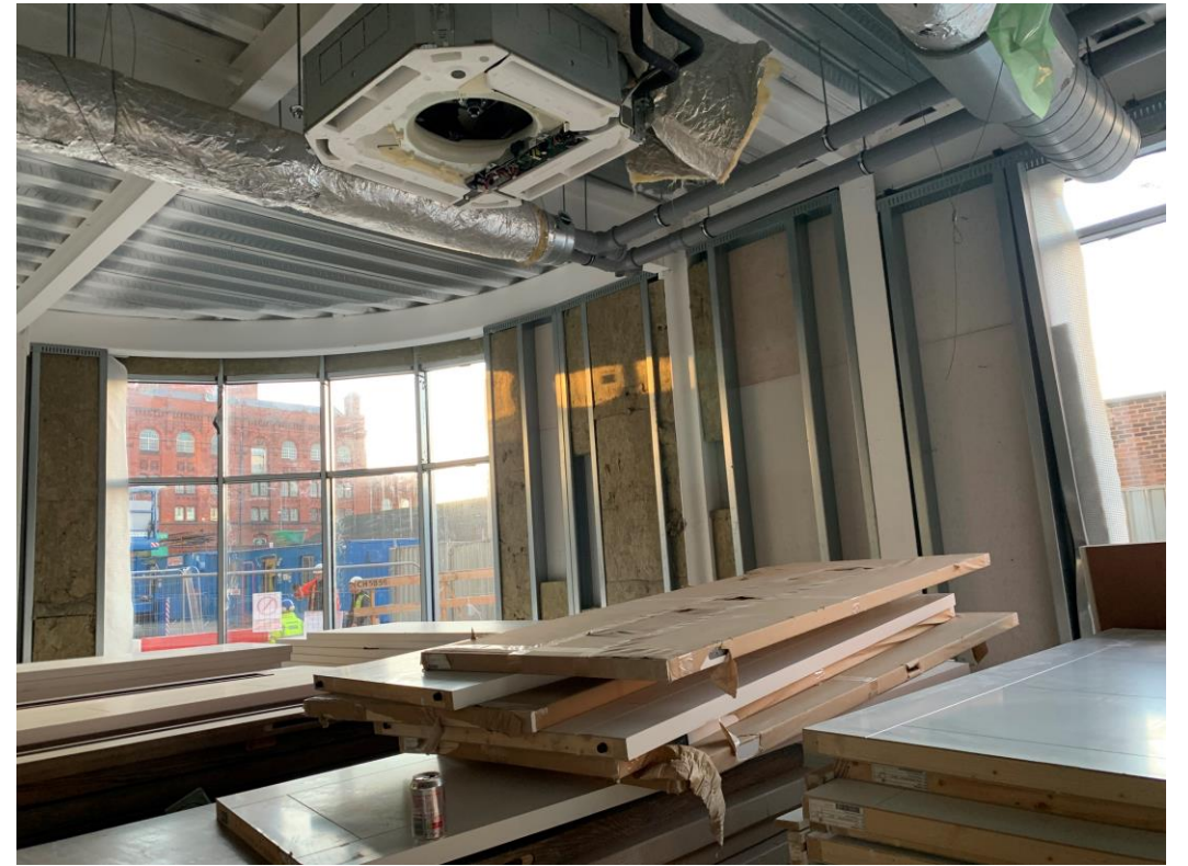
Removal of old doors ongoing
