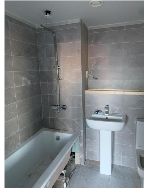
Bath, shower & WHB. Floor & wall tiling complete
