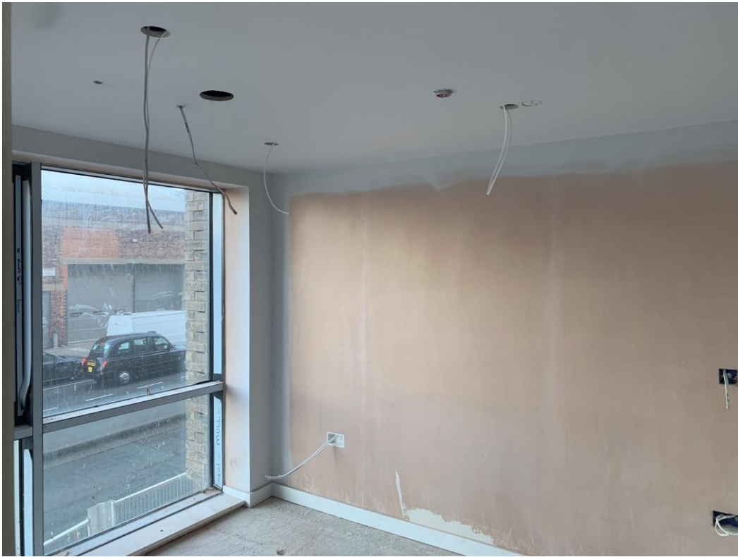
1 st Decoration coat to ceiling complete. Decoration to walls ongoing
