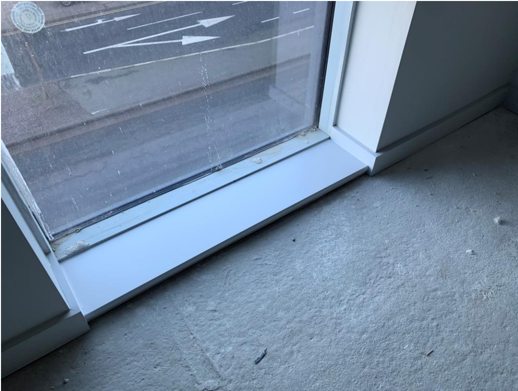
Skirting boards and window board installed
