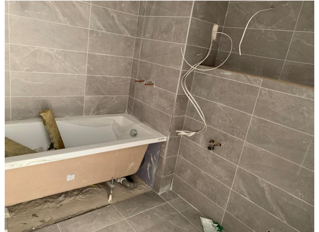
Bath installed. Floor & wall tiling complete
