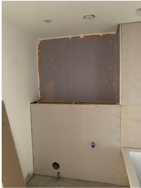
IPS boarded. Bath installed
