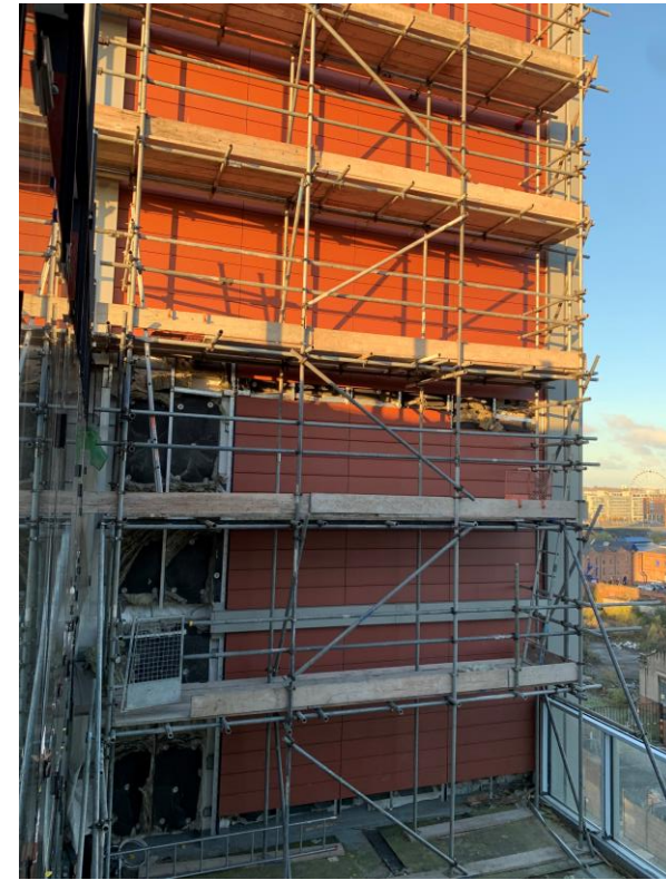
Scaffolding erected to terrace elevation. Cladding installation has commenced
