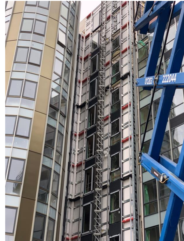
New fire barrier & cladding rail installation ongoing
