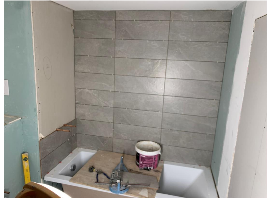
New wall tiling commenced
