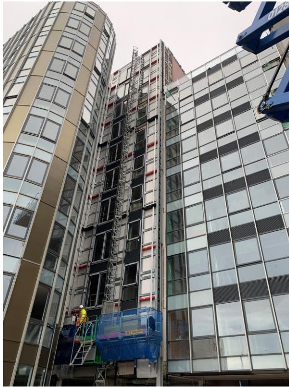
New fire barrier & cladding rail installation ongoing
