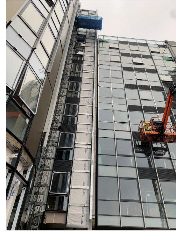
Metal grill & window trim installation ongoing
