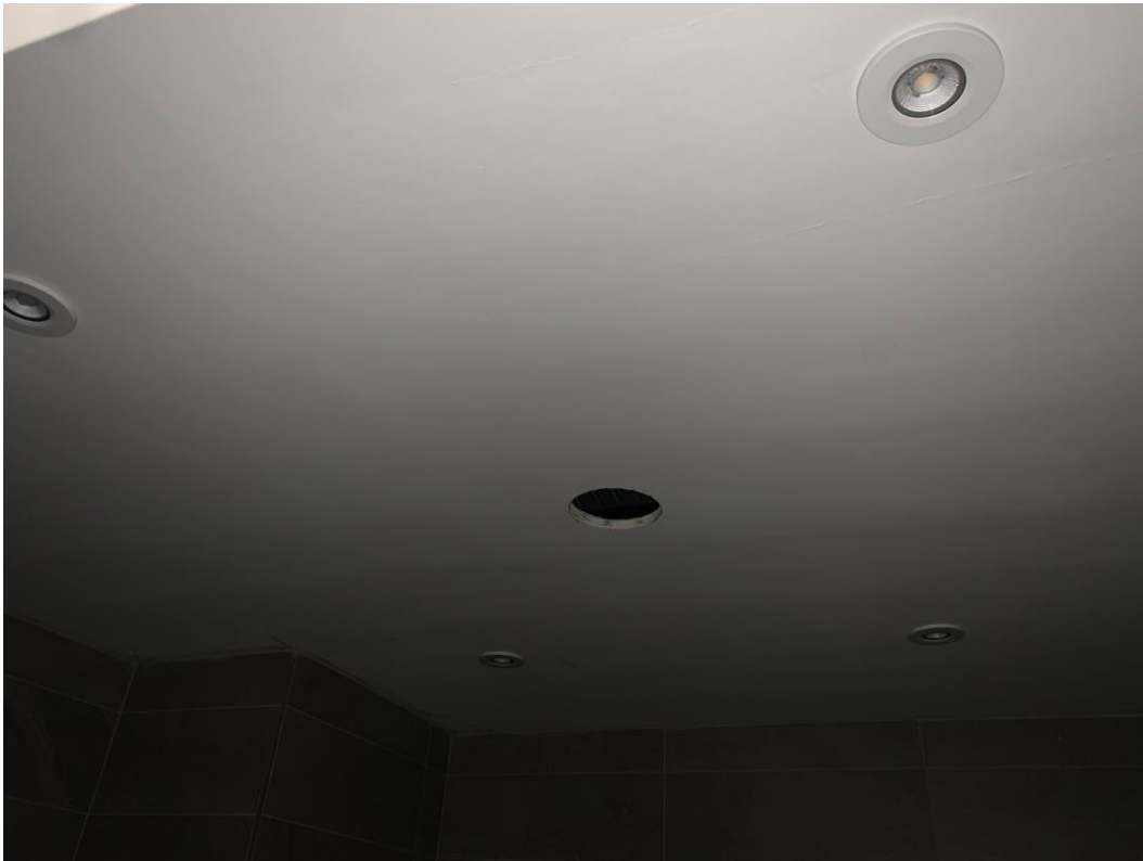
2 nd fix electric installation has commenced
