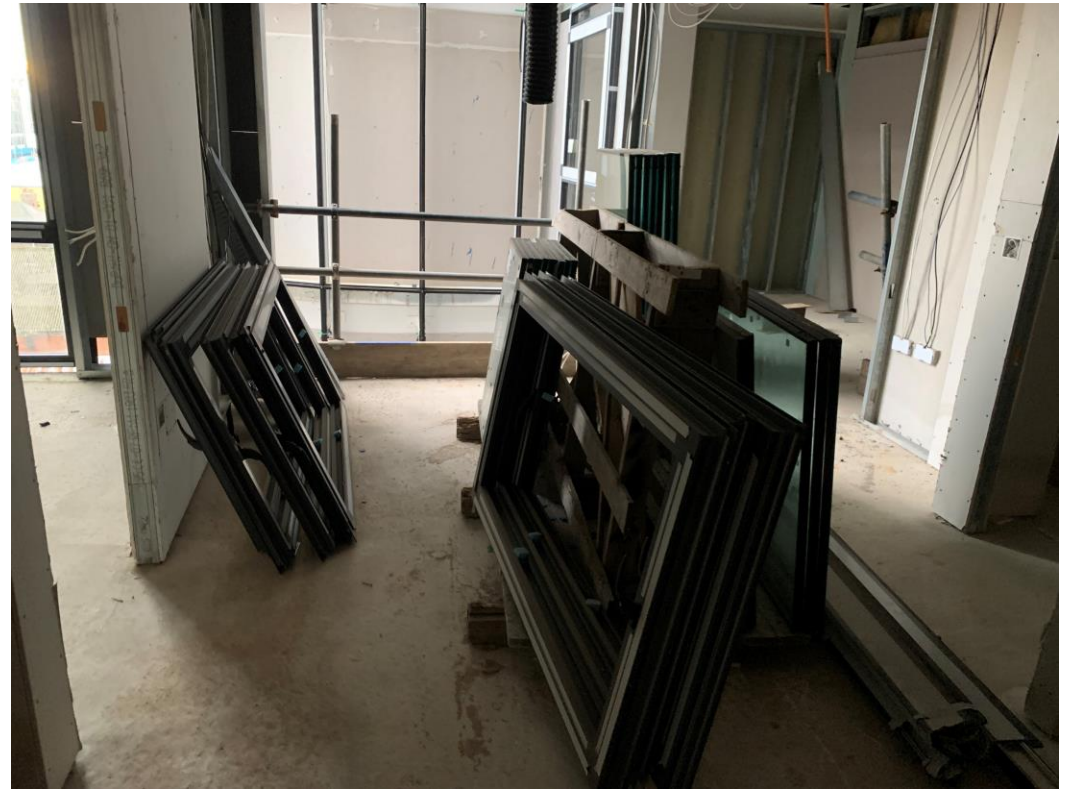
Window frames stored onsite ready for installation
