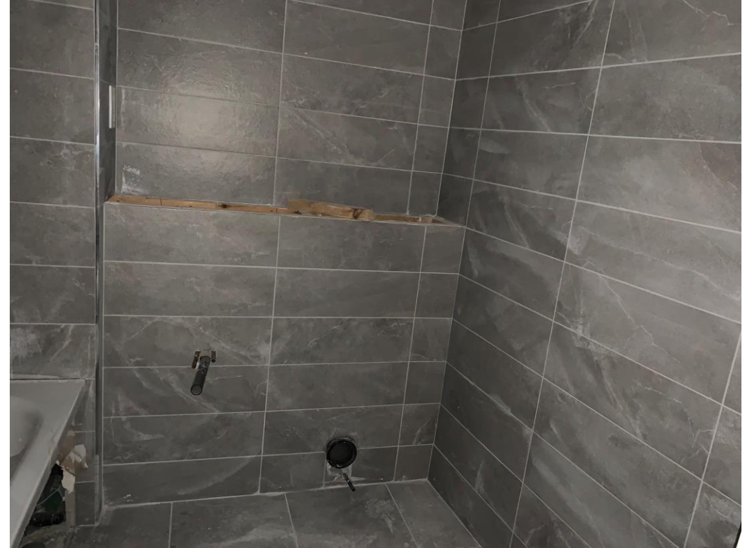
New wall & floor tile arrangement installation ongoing
