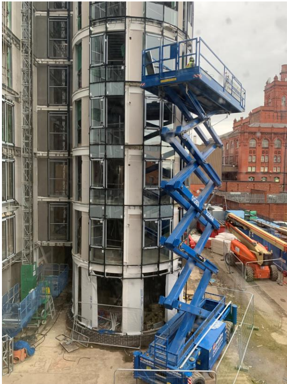
New curtain walling and glazing installation to windows ongoing
