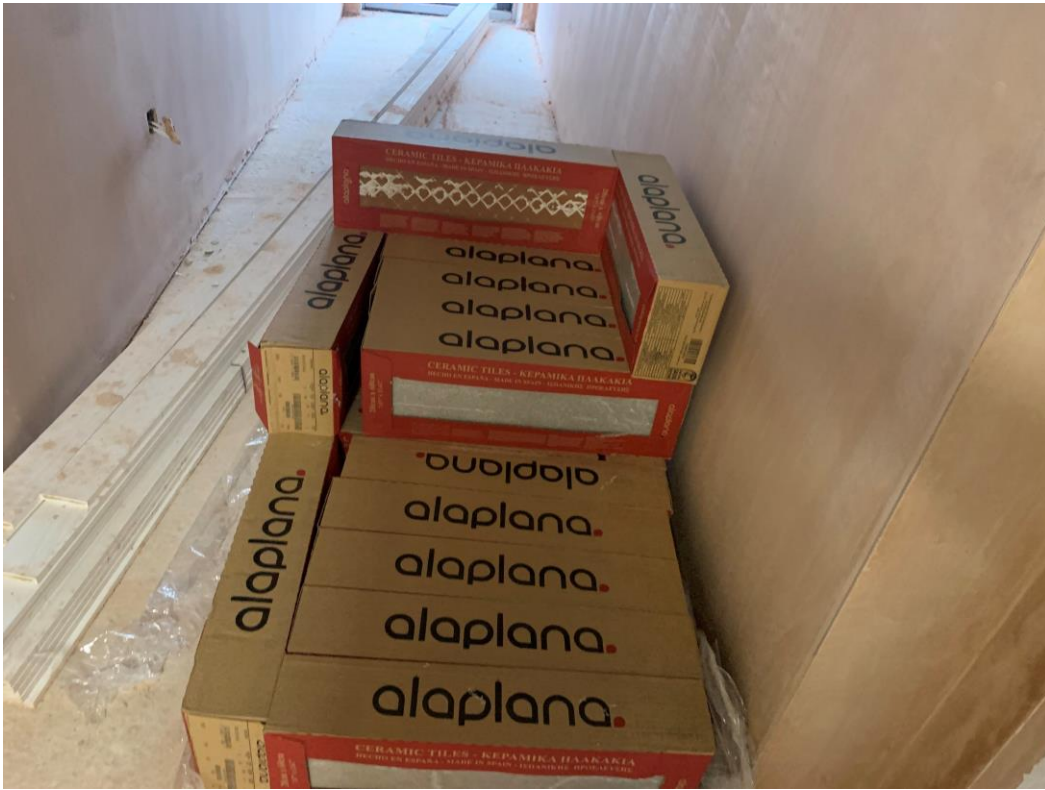
Tiles stored onsite ready for installation
