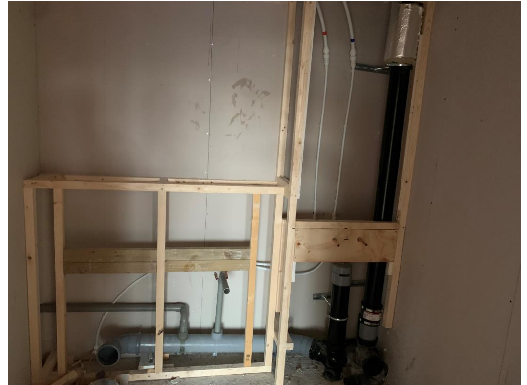
New IPS installation ongoing
