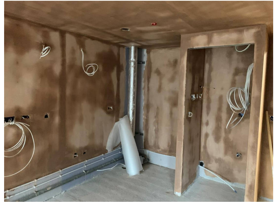
New 1 st fix electrics & plumbing. New skim of plaster
