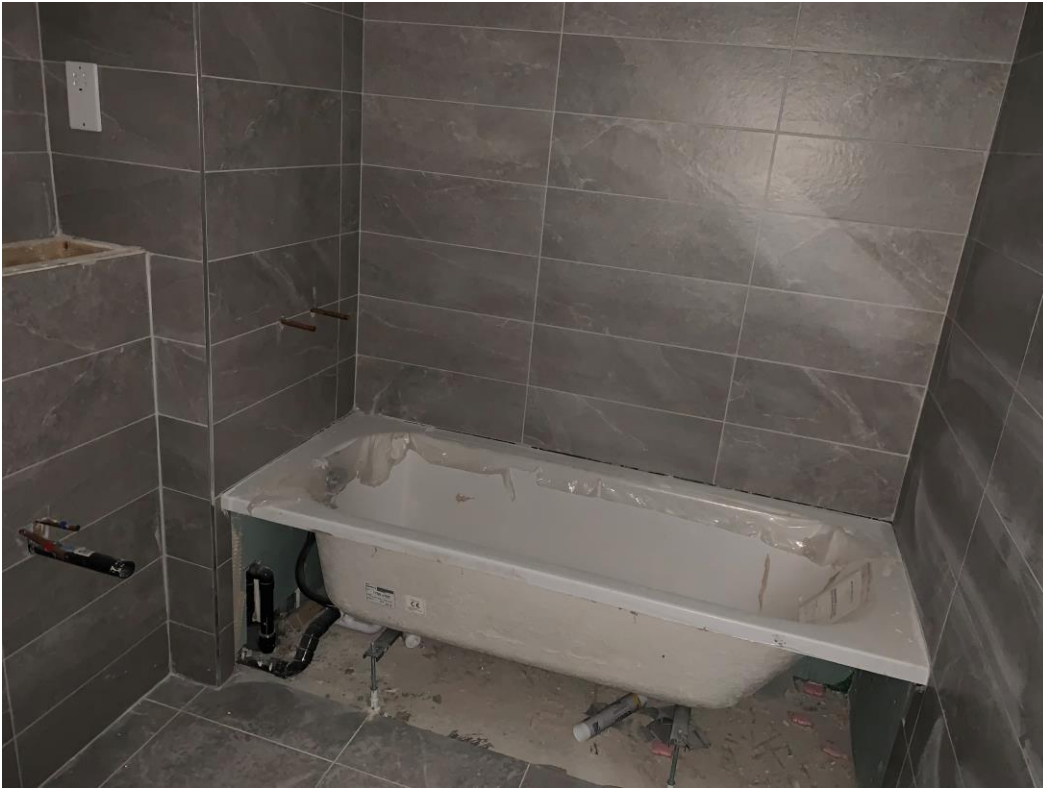
New bath & tile arrangement installation ongoing
