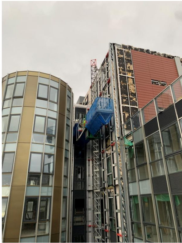
New fire barrier & cladding rail installation ongoing
