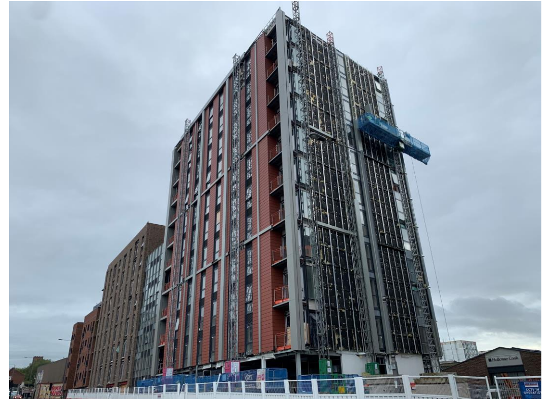
Development viewed from Parliament Street. External works ongoing
