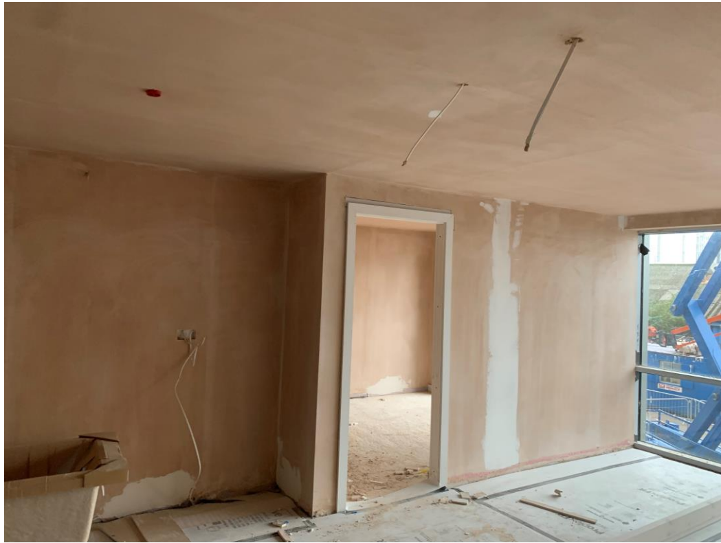
Door Linings, skirting board & architrave installation has commenced
