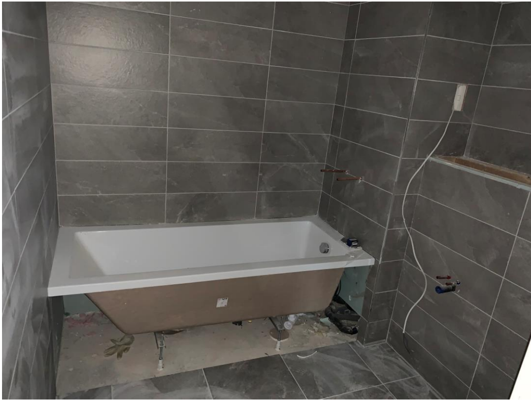
New bath & tile arrangement installation ongoing
