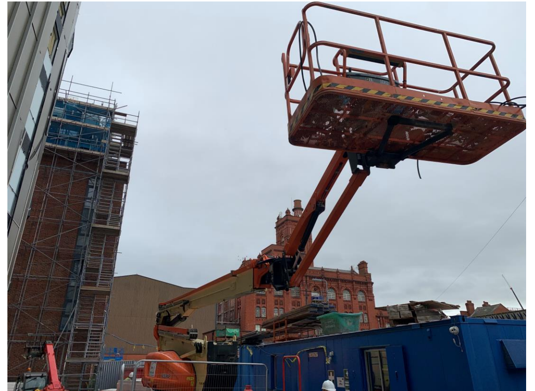
Cherry picker on site
