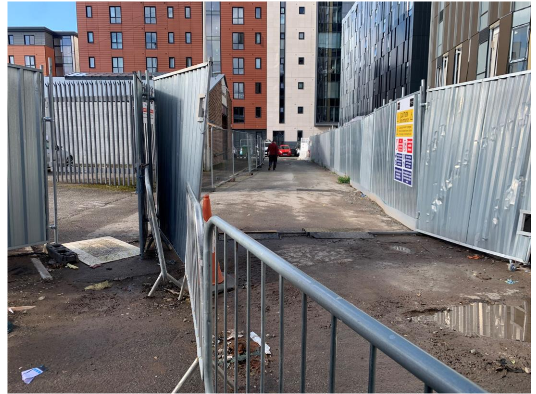
Site access from Brindley Street
