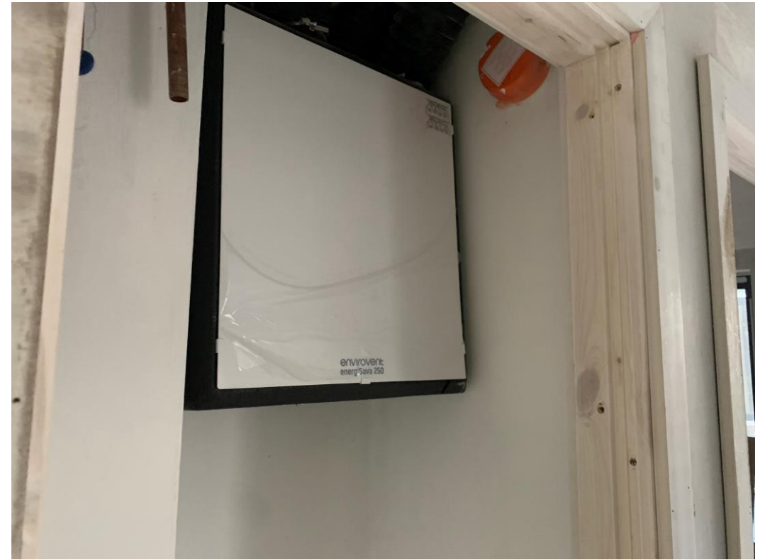
New heating ventilation system installation commenced
