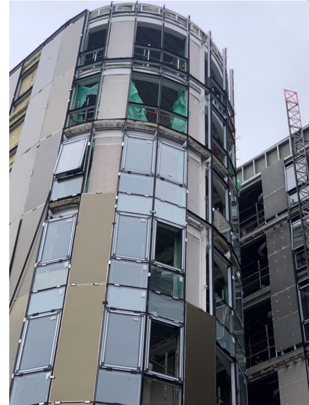
New curtain walling installation ongoing. Glazing installation ongoing
