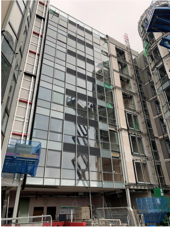
Metal grill & window trim installation ongoing
