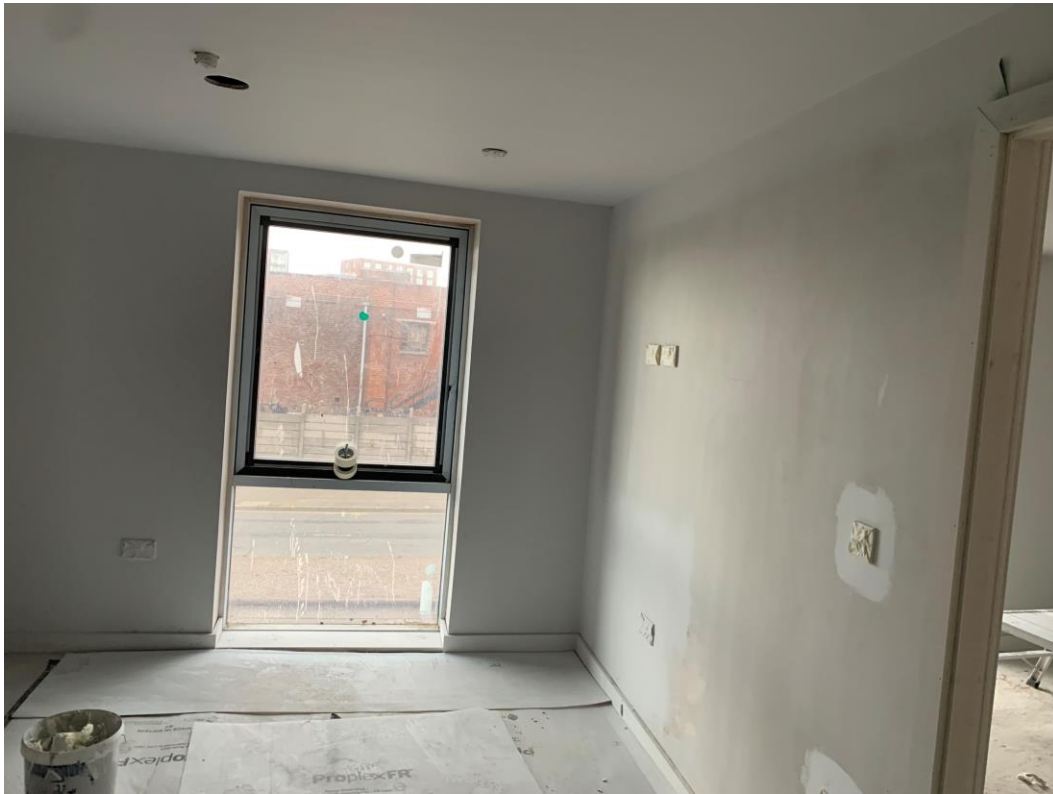
Ceilings and walls 1 st decoration coat. Floor finishes installed & protected
