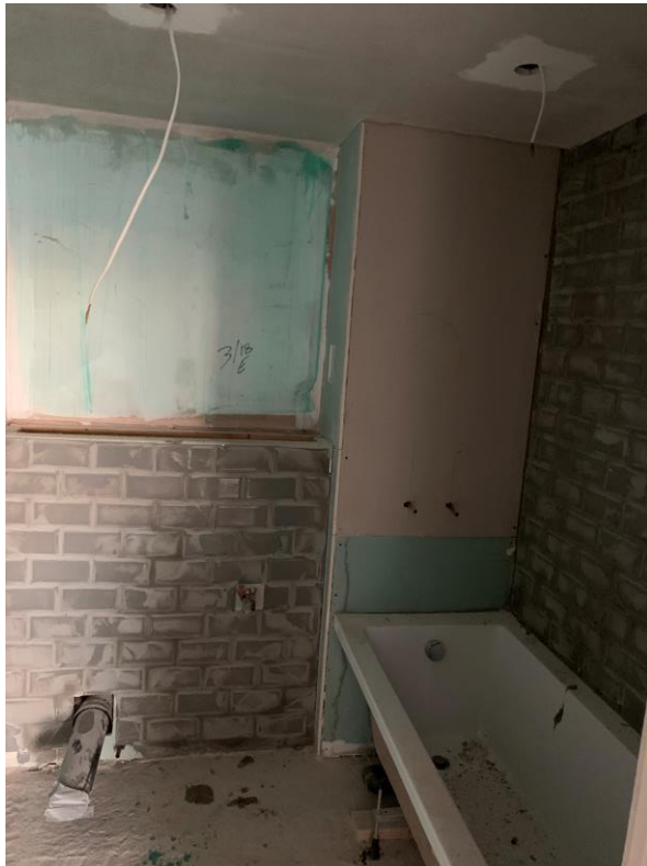
Replacement bath fittings installed and prepped for tiling
