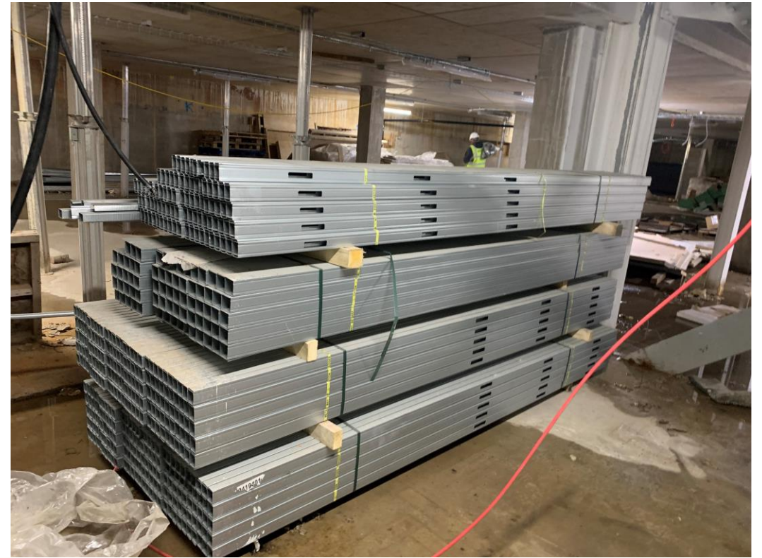
Metal partition material store onsite ready for installation
