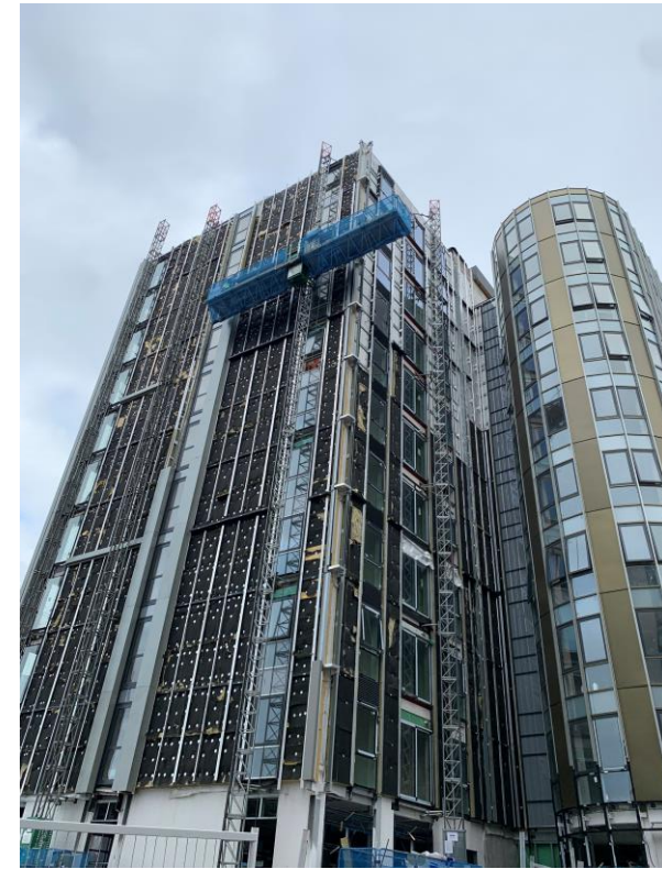
Development viewed from Caryl Street. External works ongoing
