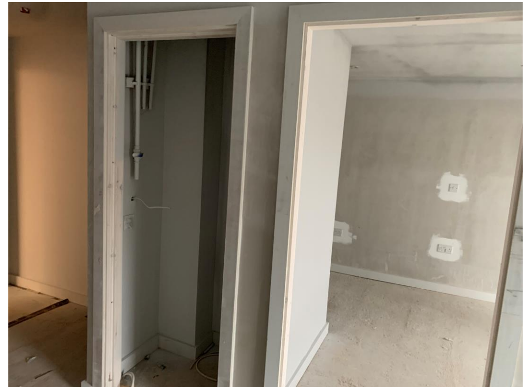
Door linings, skirting boards & architrave installation has commenced
