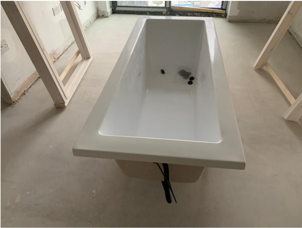
Baths stored onsite ready for installation
