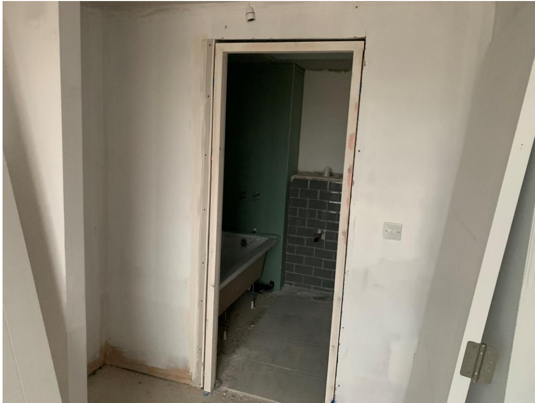
Door linings installation has commenced
