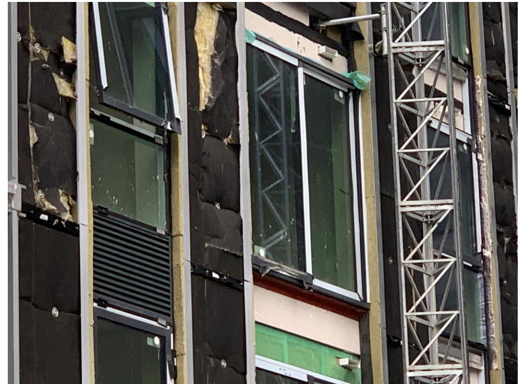
Cladding removal & insulation installation ongoing. Installation of new balcony doors ongoing
