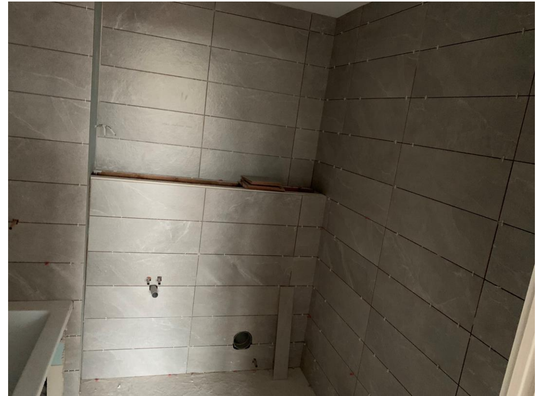
New vanity tile arrangement installation ongoing
