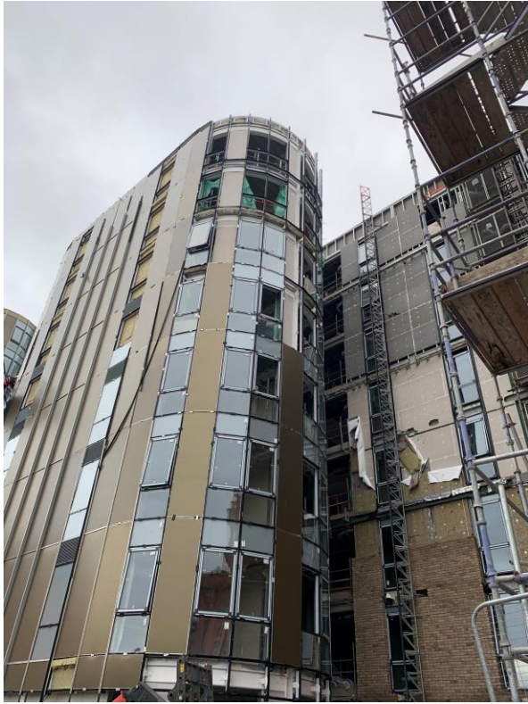
New curtain walling installation ongoing. Glazing installation ongoing
