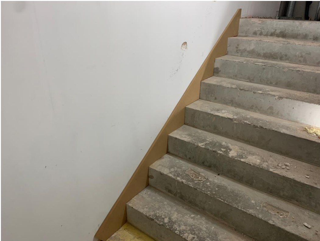
New stringer installation has commenced
