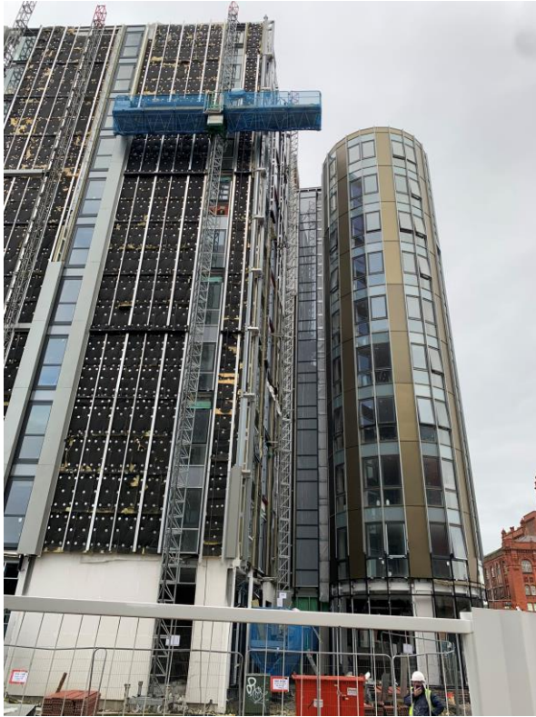
Development viewed from Caryl Street. External works ongoing
