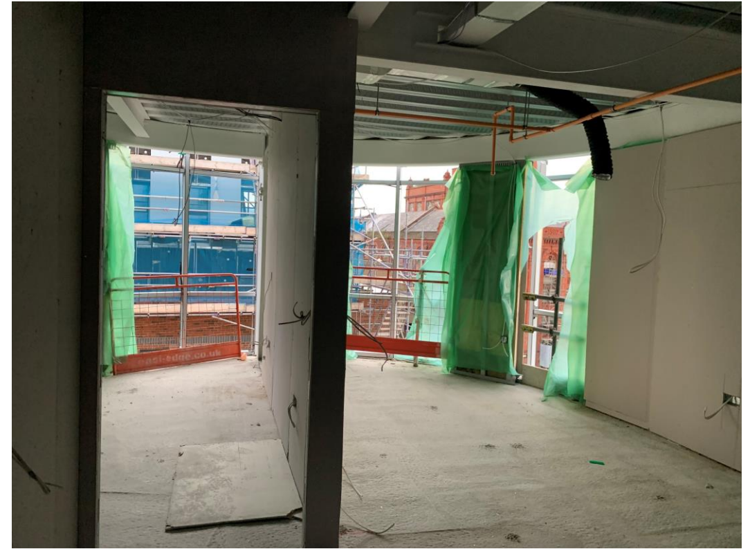
Glazing installation ongoing
