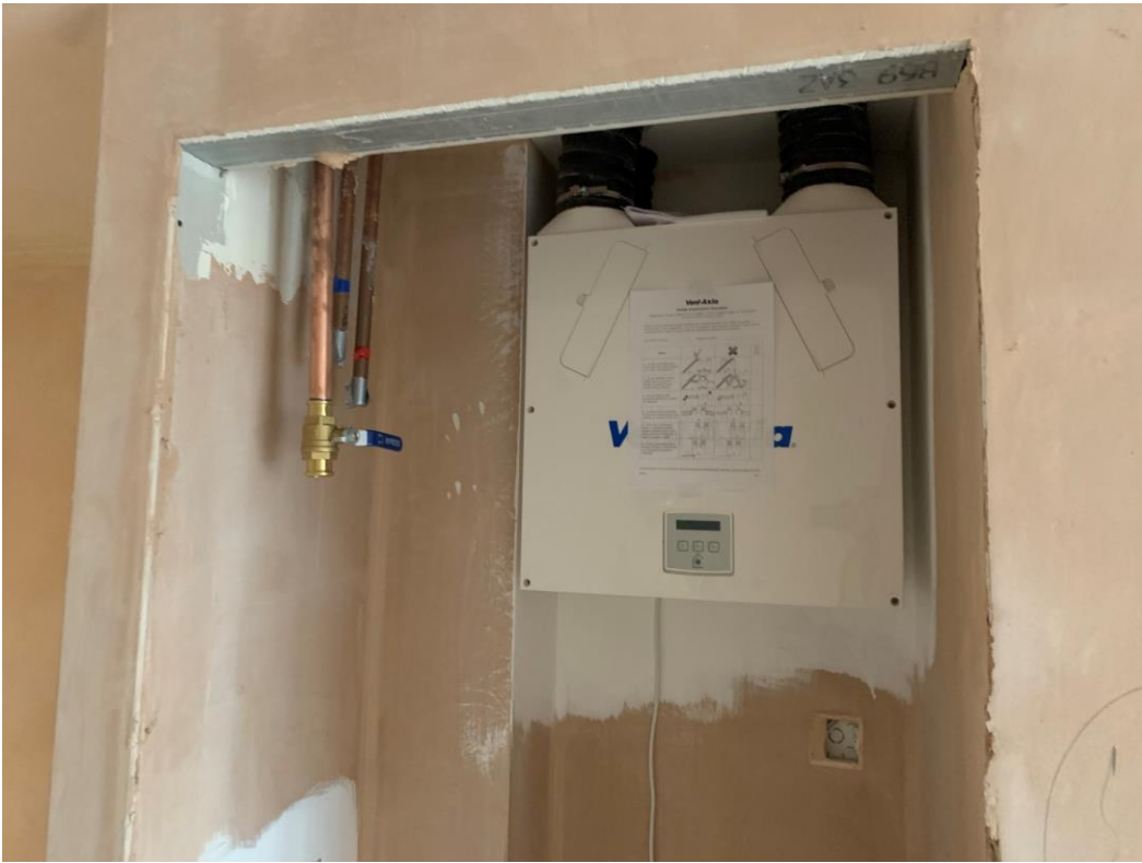
Old heating ventilation system
