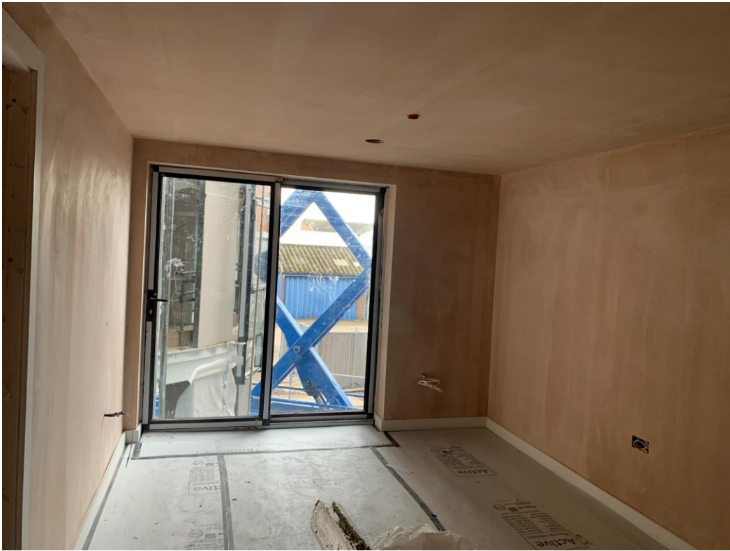
New skim of plaster to lounge area of apartments
