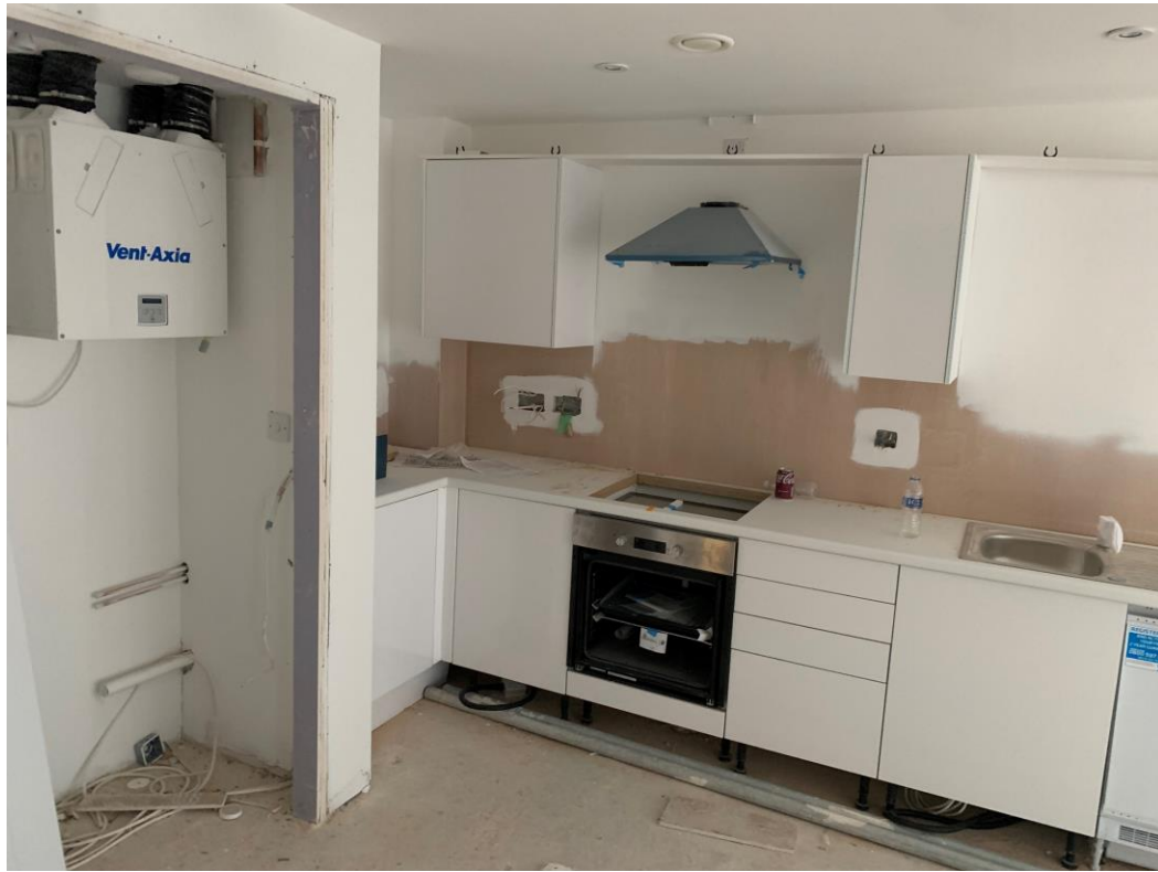
Old Kitchen and boiler, prior to removal
