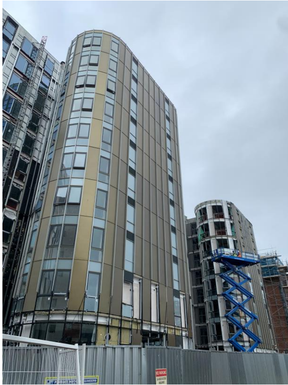
External cladding remedial works and reinstated
