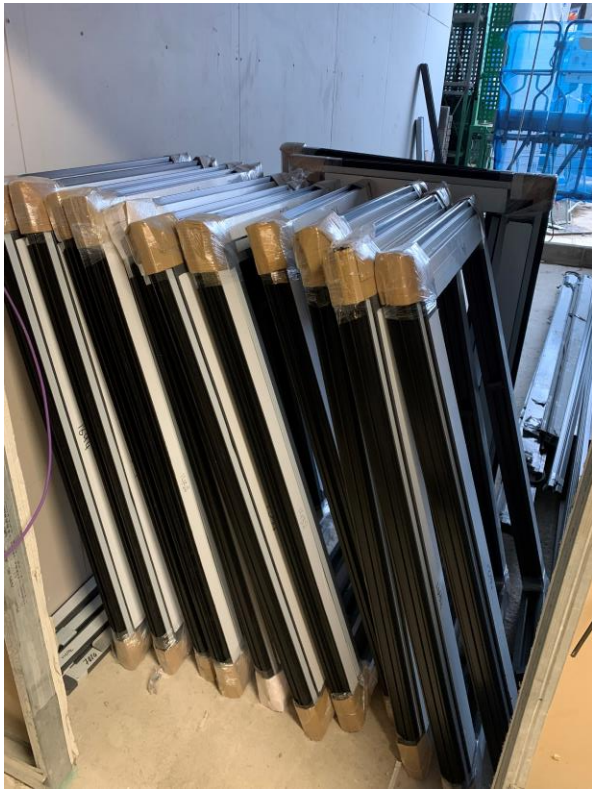
Window frames stored onsite ready for installation
