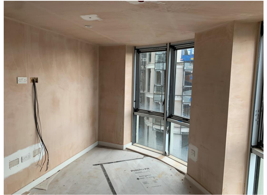
New skim of plaster to lounge area of apartment
