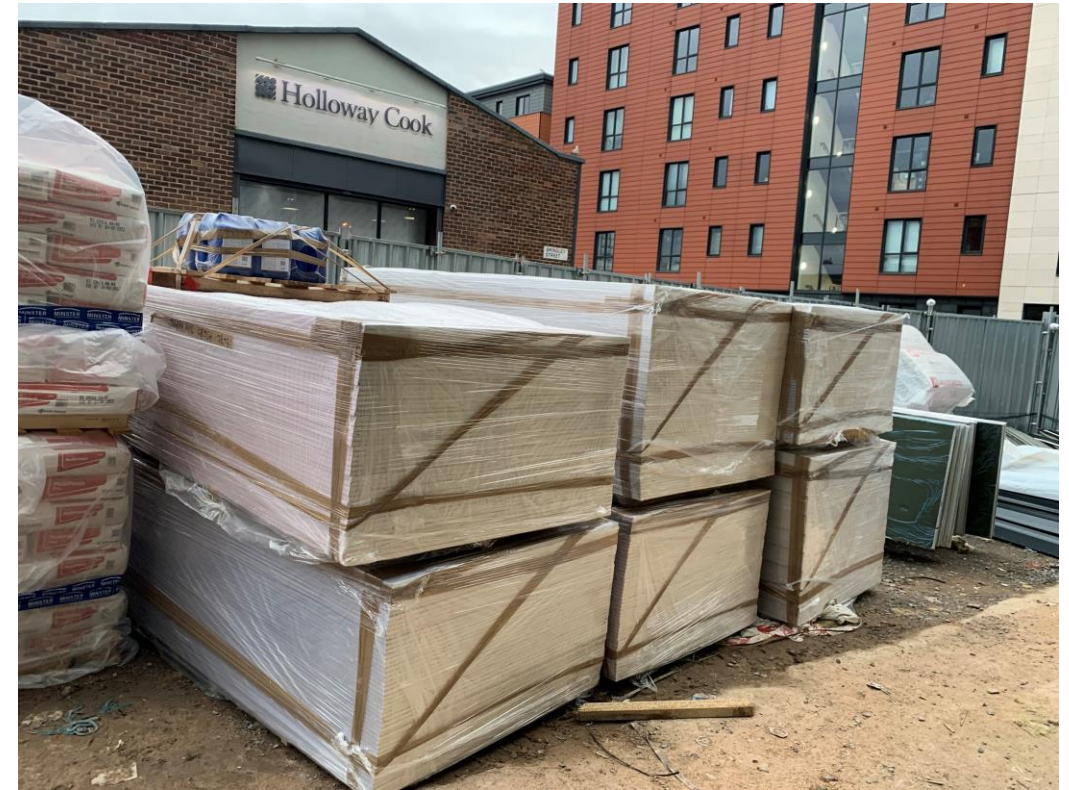
Site material storage
