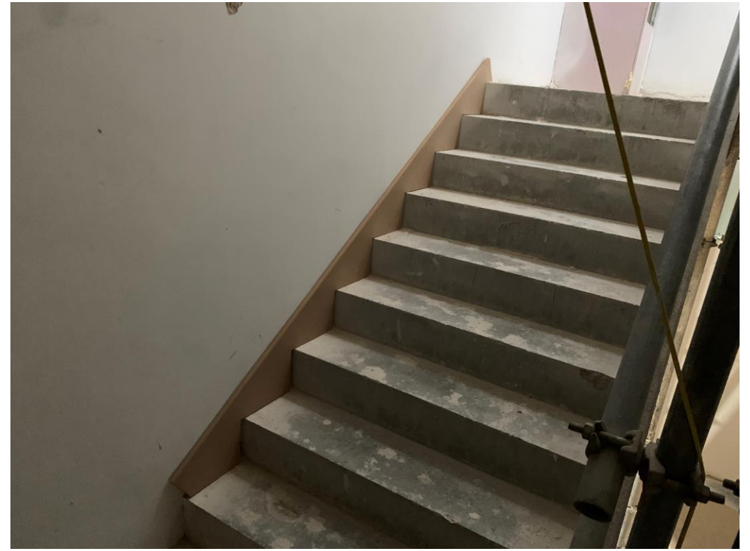
New stringer installation has commenced
