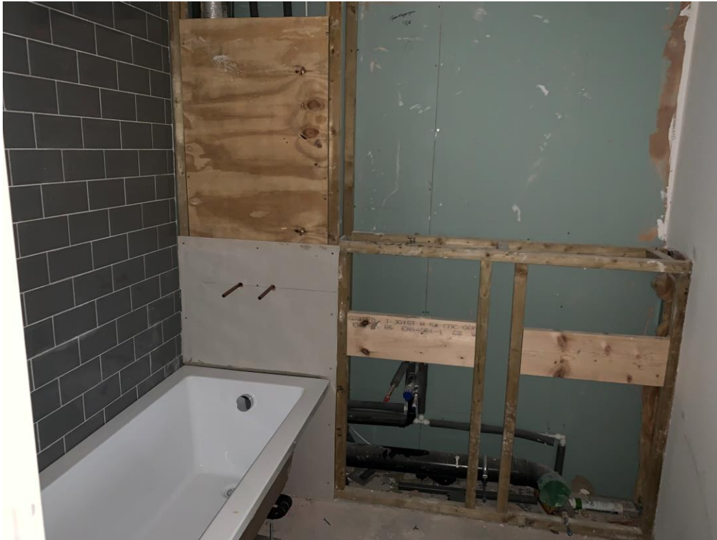
Replacement bath fittings installed and prepped for tiling
