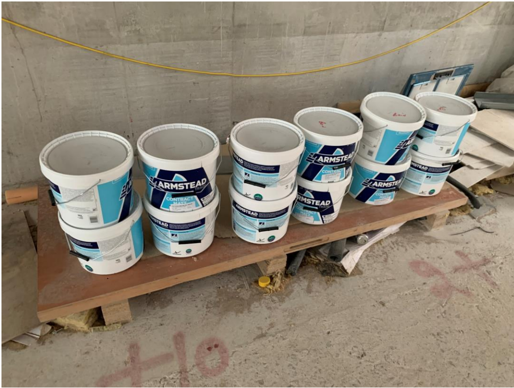
Material stored onsite ready for application
