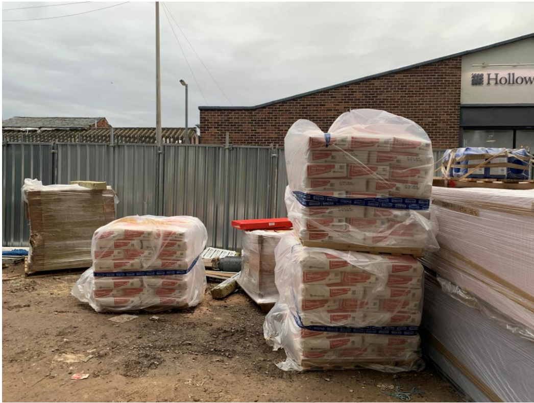
Site material storage
