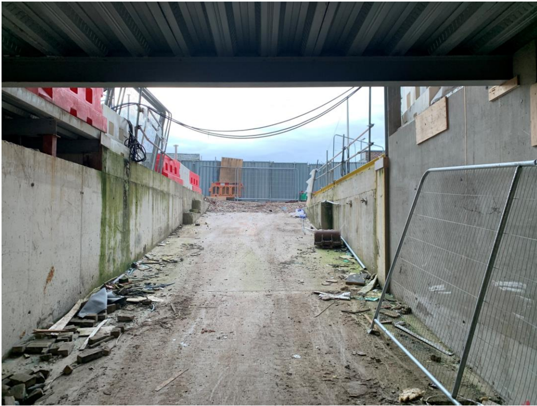
Ramp leading into basement
