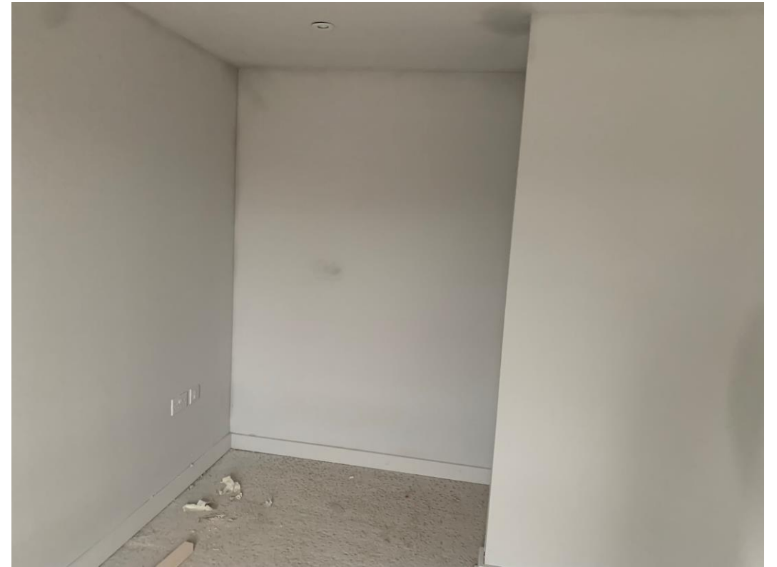
Ceilings and walls 1 st decoration coat
