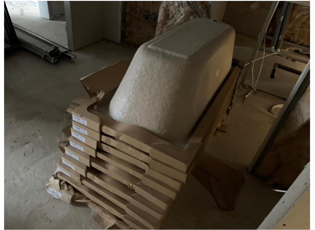
Baths stored onsite ready for installation
