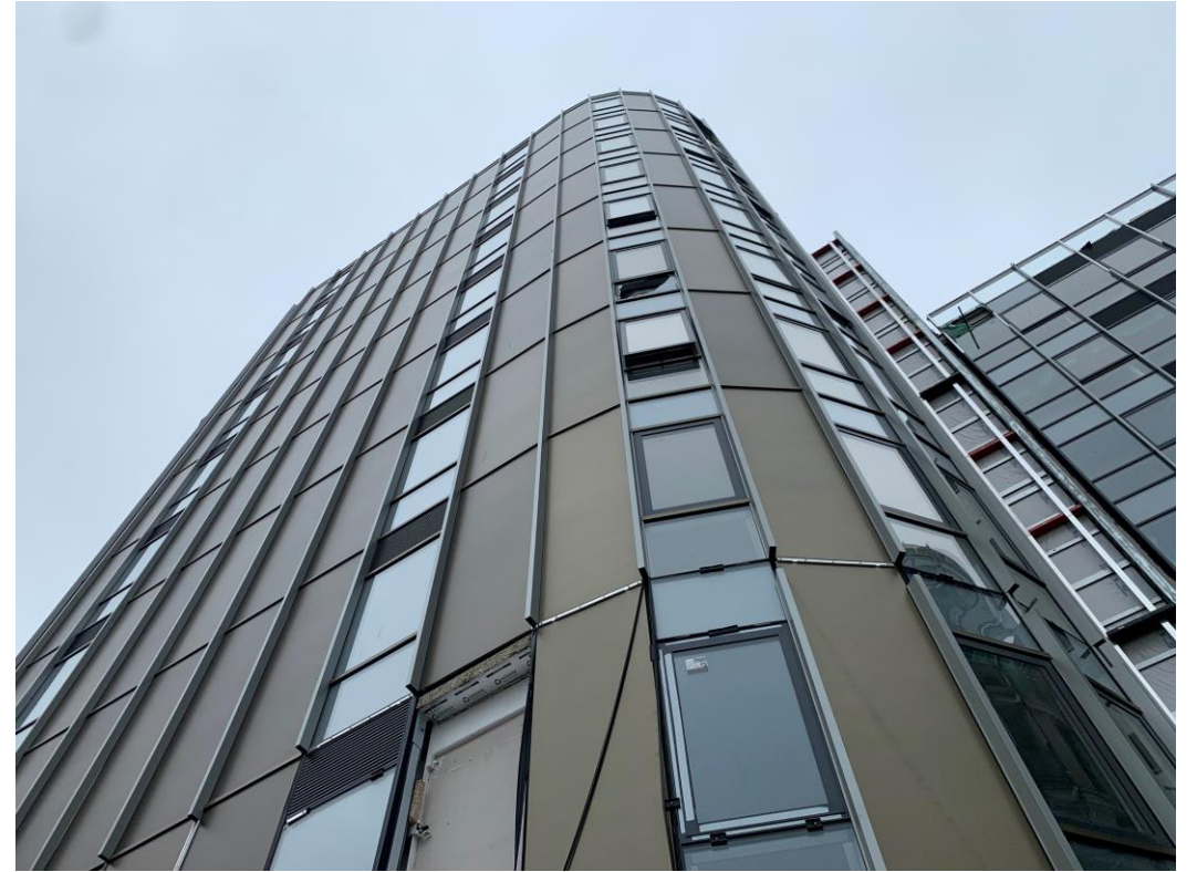
External cladding remedial works and reinstated
