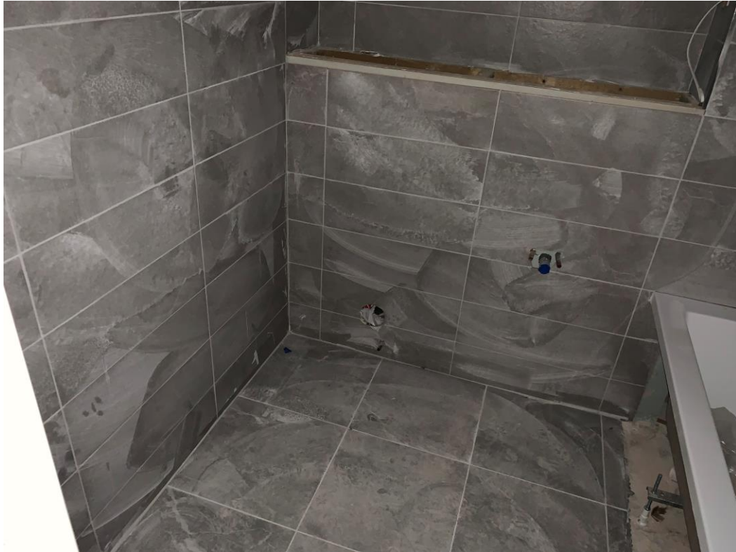
New wall & floor tile arrangement installation ongoing
