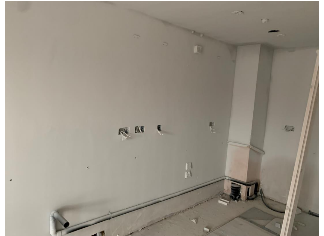
1 st fix electrics & plumbing. 1 st coat of paint
