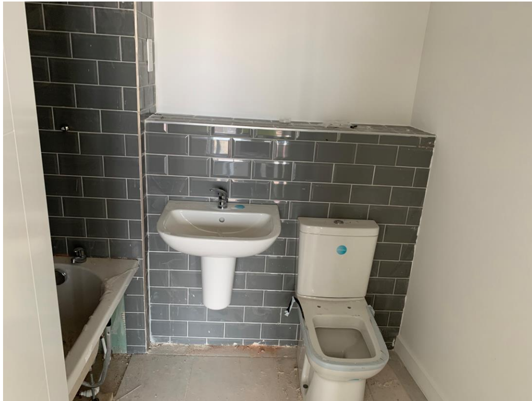
Old bathroom sanitary fittings & tiling
