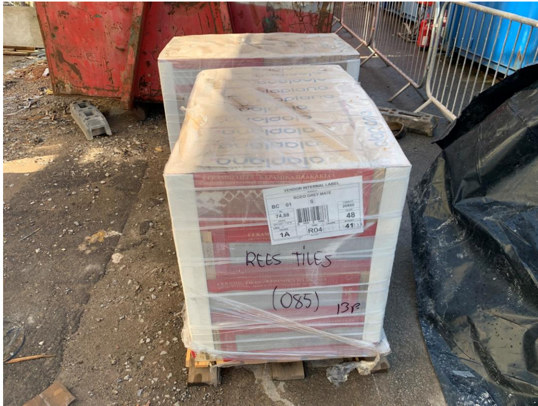
Site material storage
