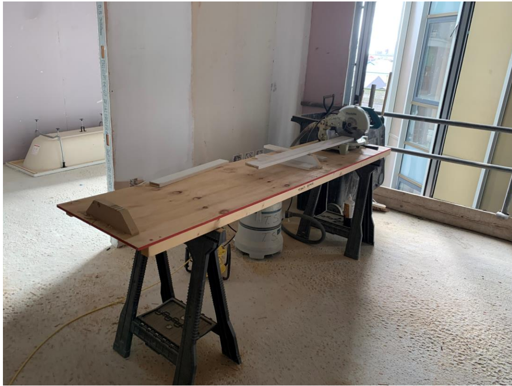
New skirting boards and architrave being installed
