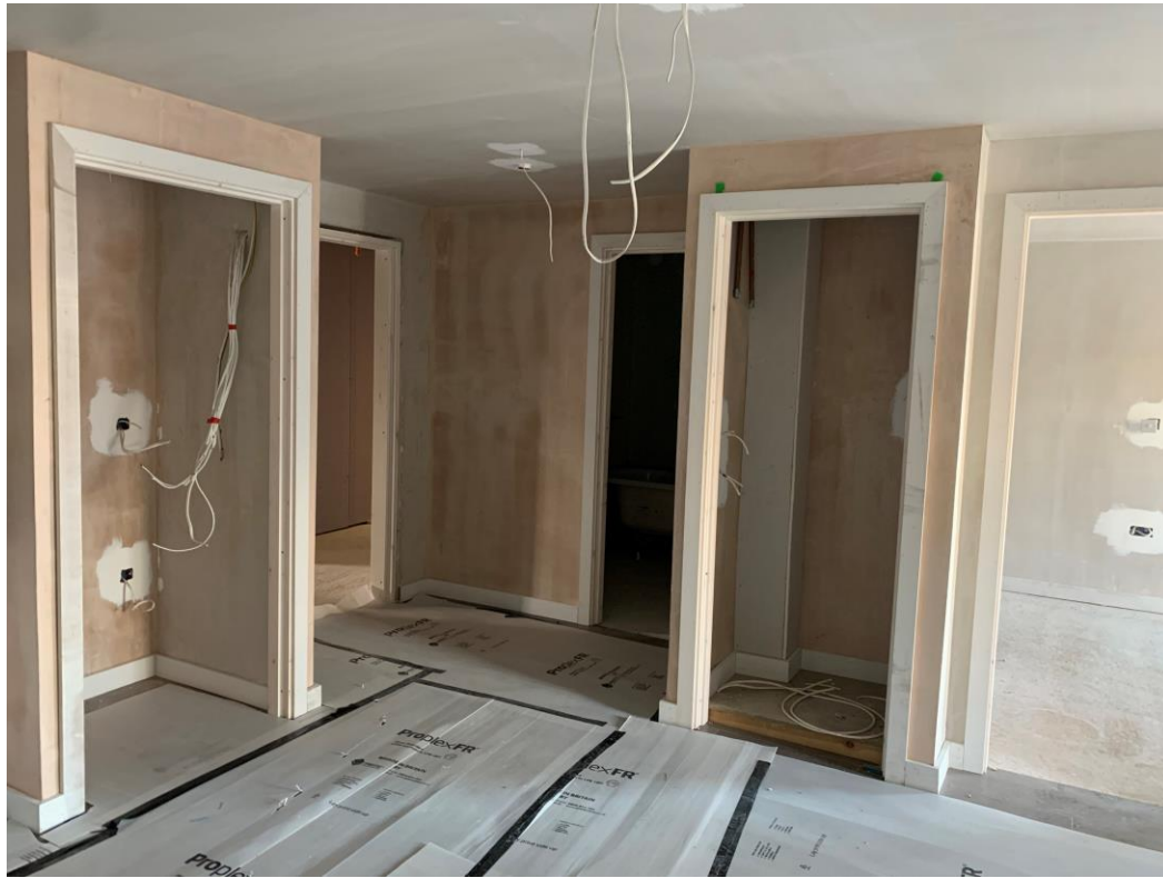
Floor finishes installed & protected
