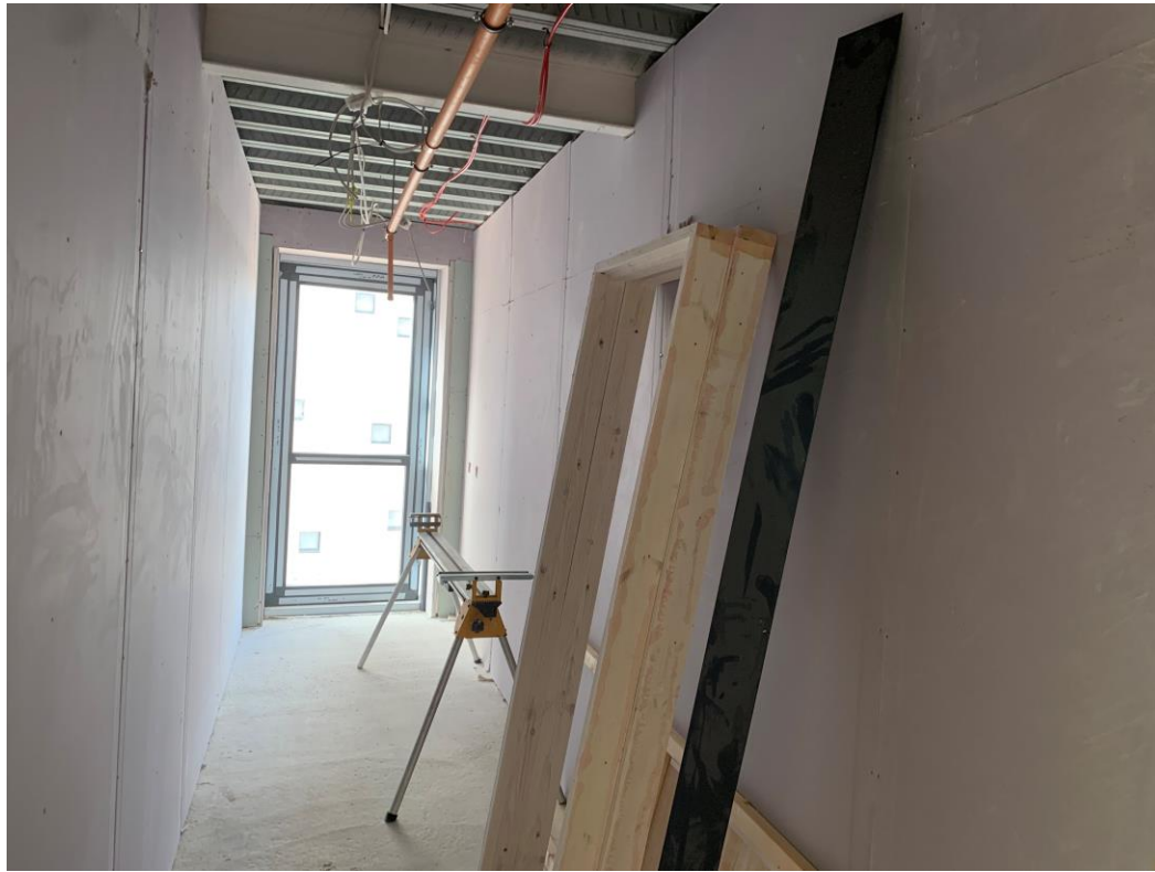
New doorframe being installed
