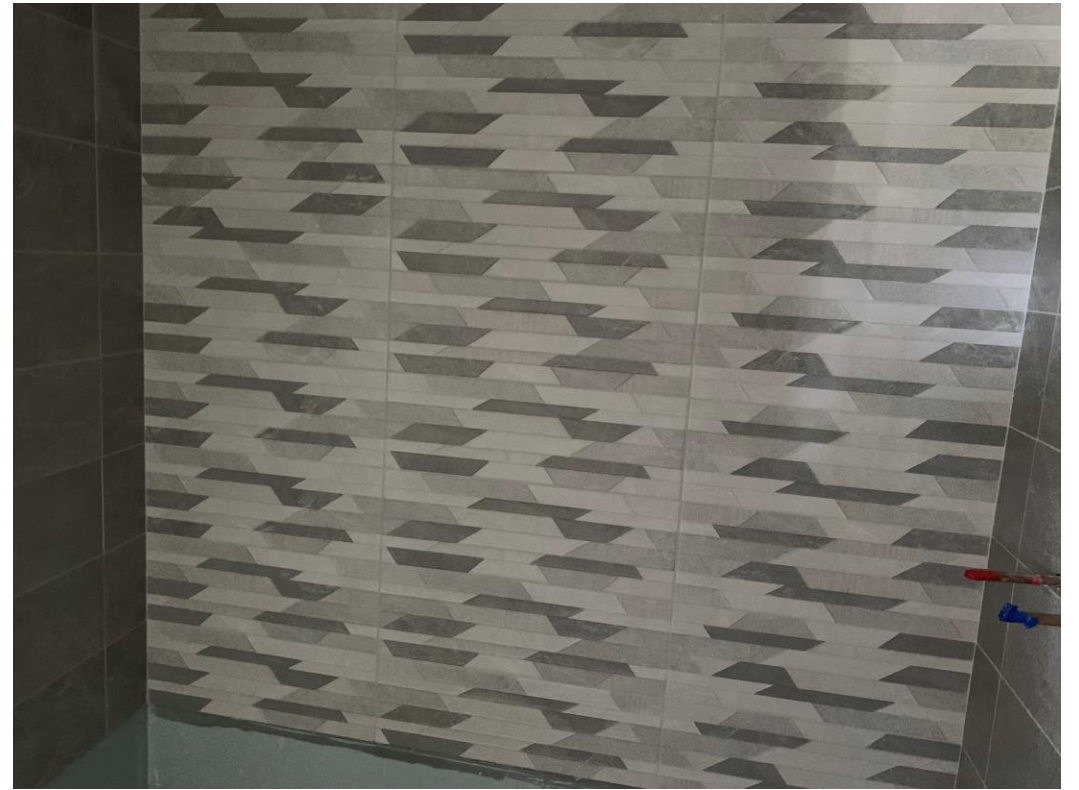
New bathroom tiling sample for shower area
