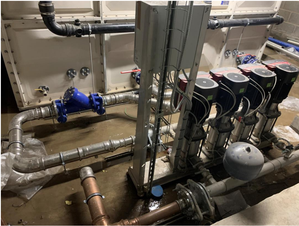
Basement Plant room fit out ongoing
