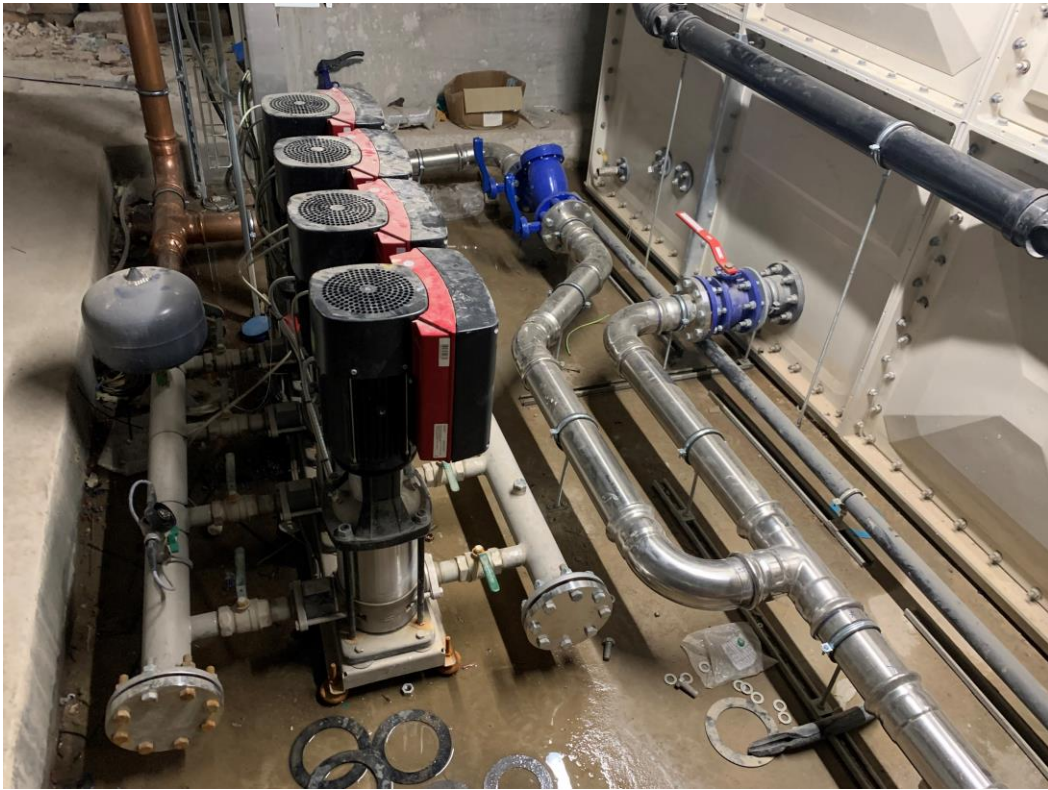
Basement Plant room fit out ongoing
