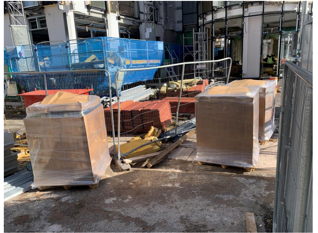
Site material storage
