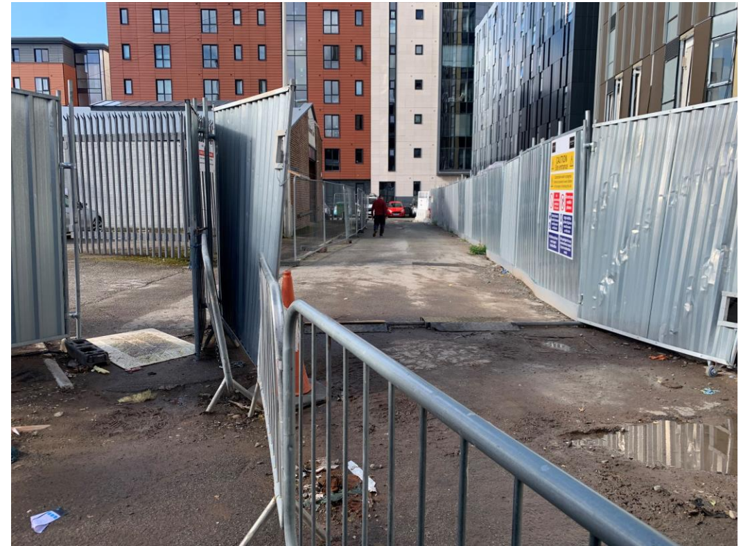
Site access from Brindley Street
