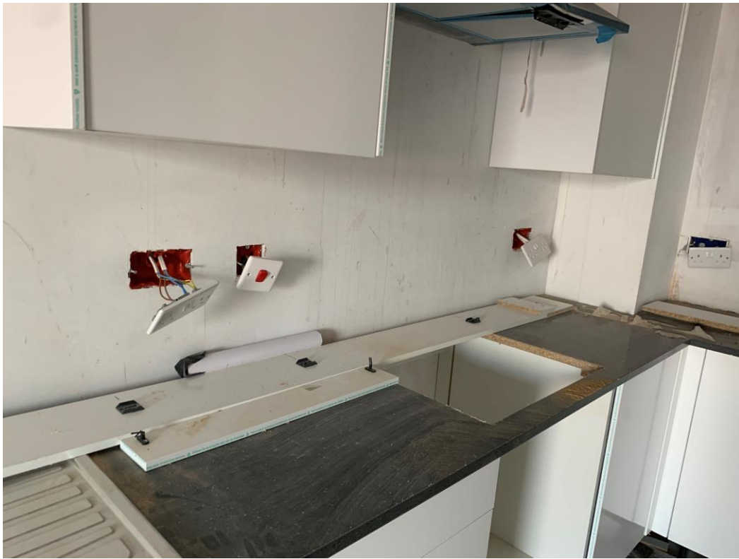
Kitchen removal ongoing
