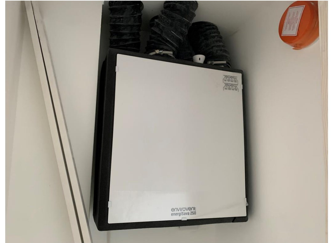
Mechanical ventilation installed / kitchen commenced
