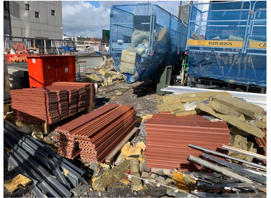
Site material storage
