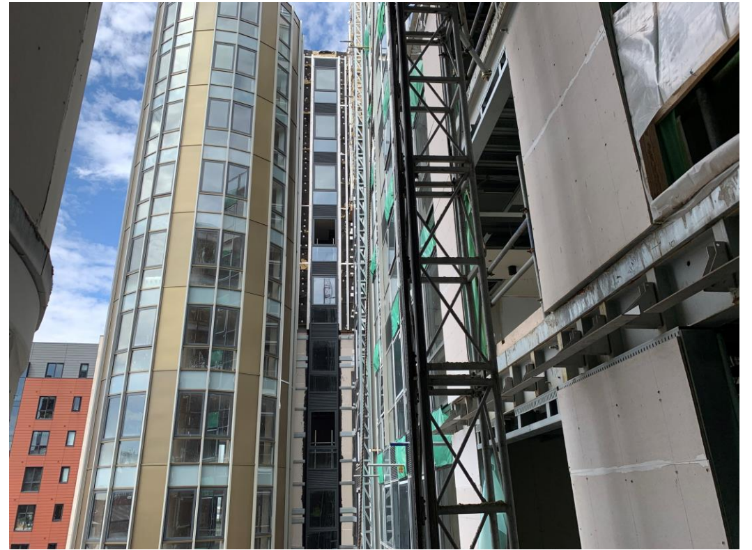
External cladding installed
