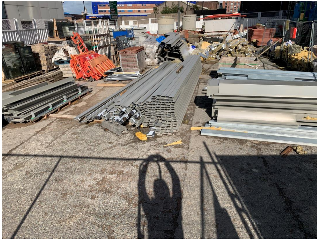
Cladding material storage
