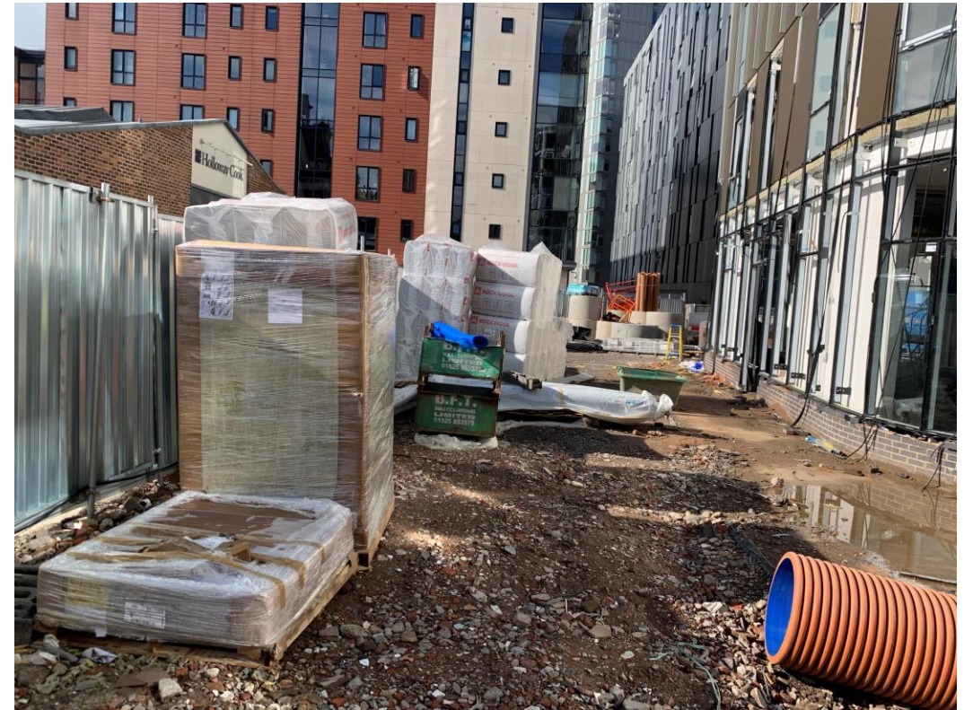
Site material storage
