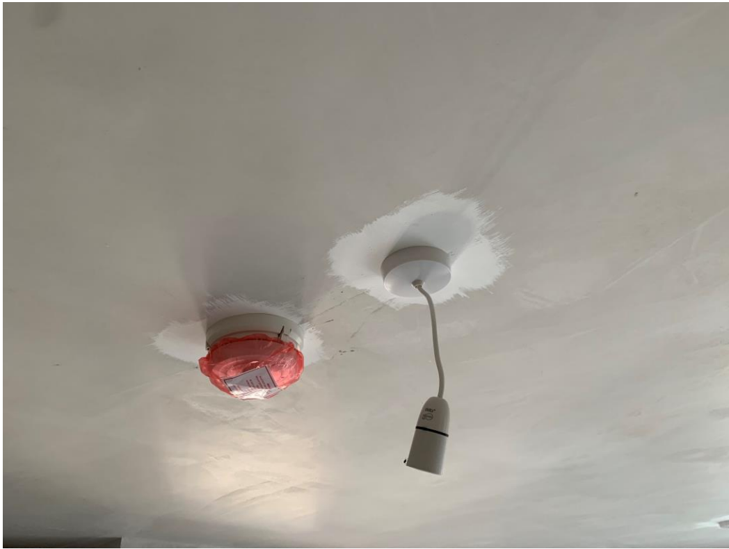
2 nd Smoke detection and lighting ongoing
