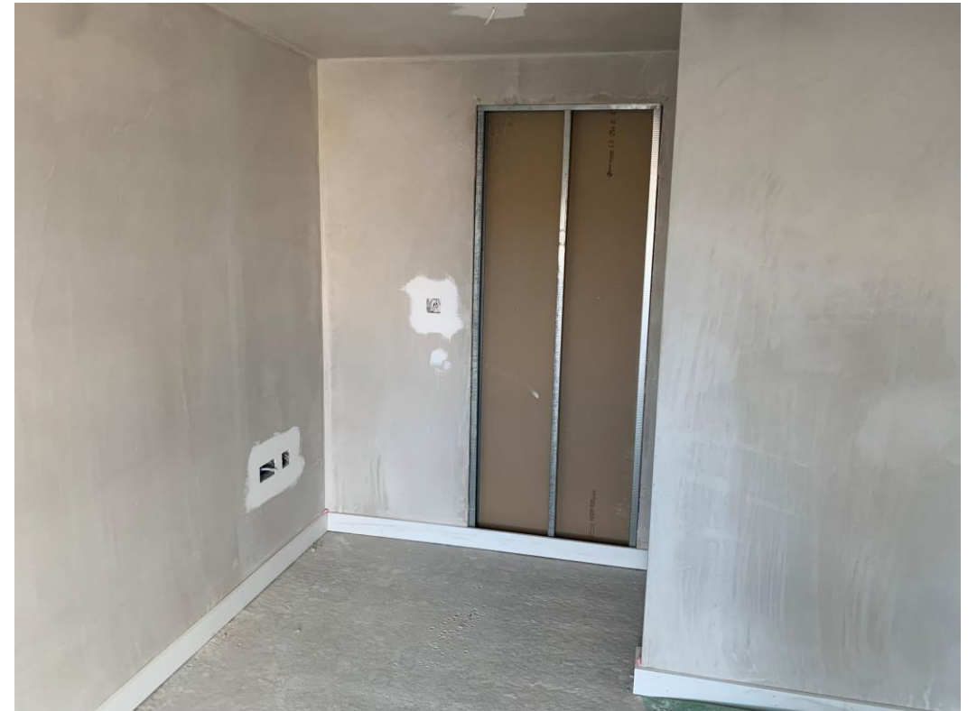
Jack & Gill bathroom door removed and boarded on the bedroom side
