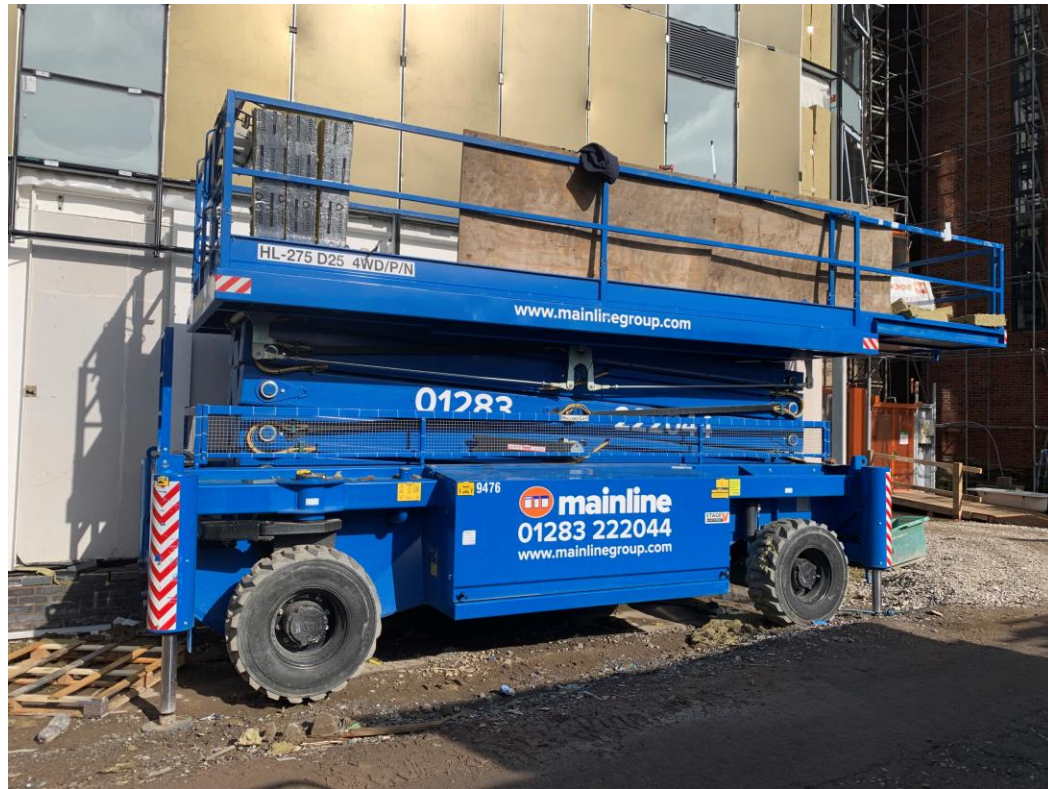
Scissor lift onsite
