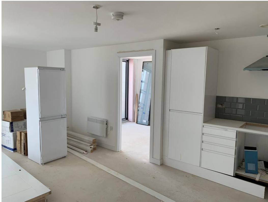
Lounge area prior to floor installation
