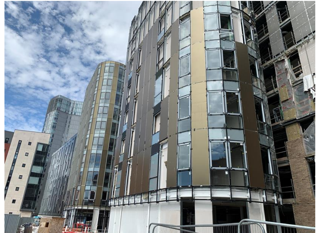
Development viewed from Caryl Street. Cladding pre inspection.
