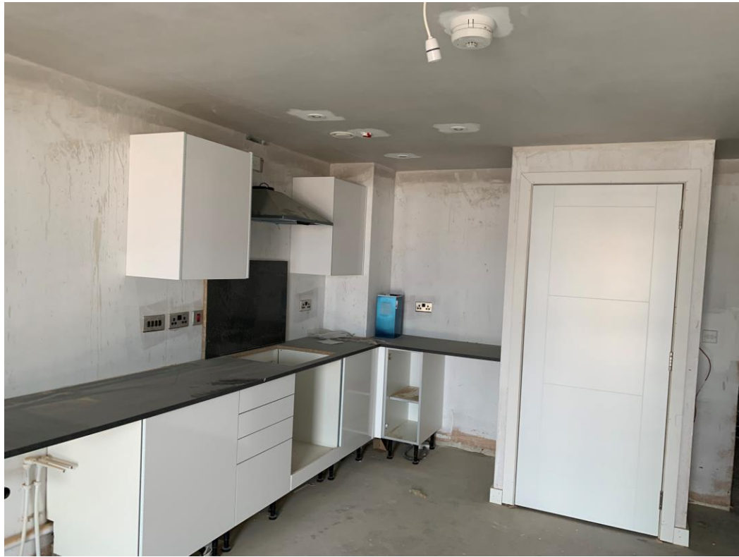
Old Kitchen and boiler door, prior to removal
