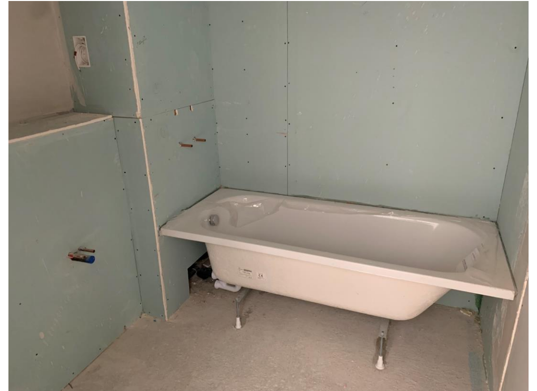
New bathroom sanitary fitting installation ongoing
