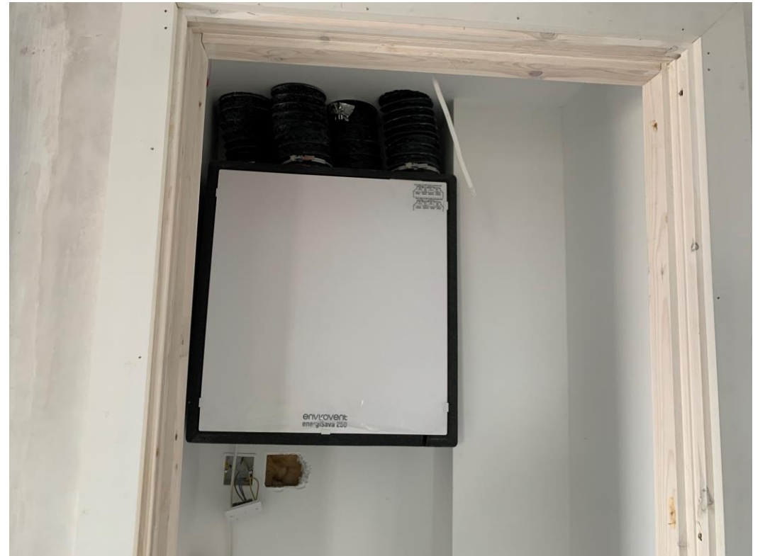
Replacement mechanical heat ventilation installed
