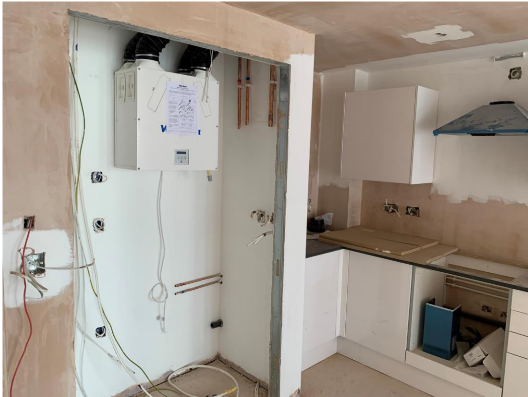
Mechanical ventilation & water cylinder installed
