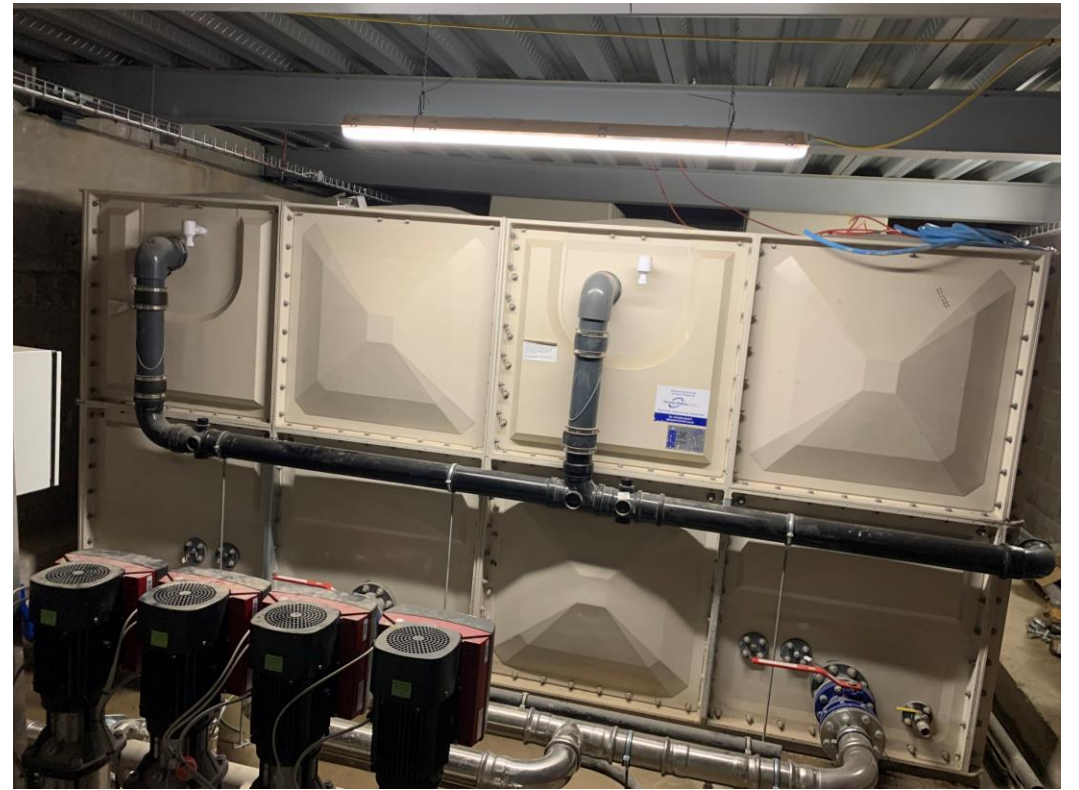
Basement Plant room fit out ongoing
