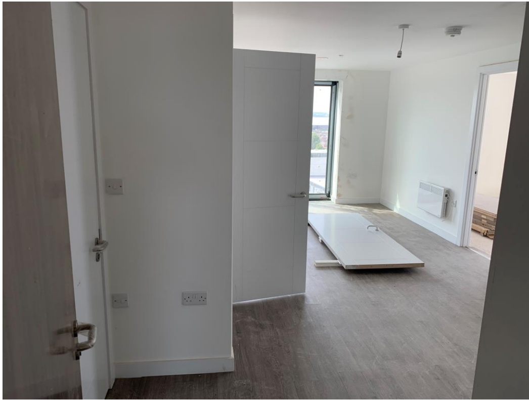
Old doors prior to removal
