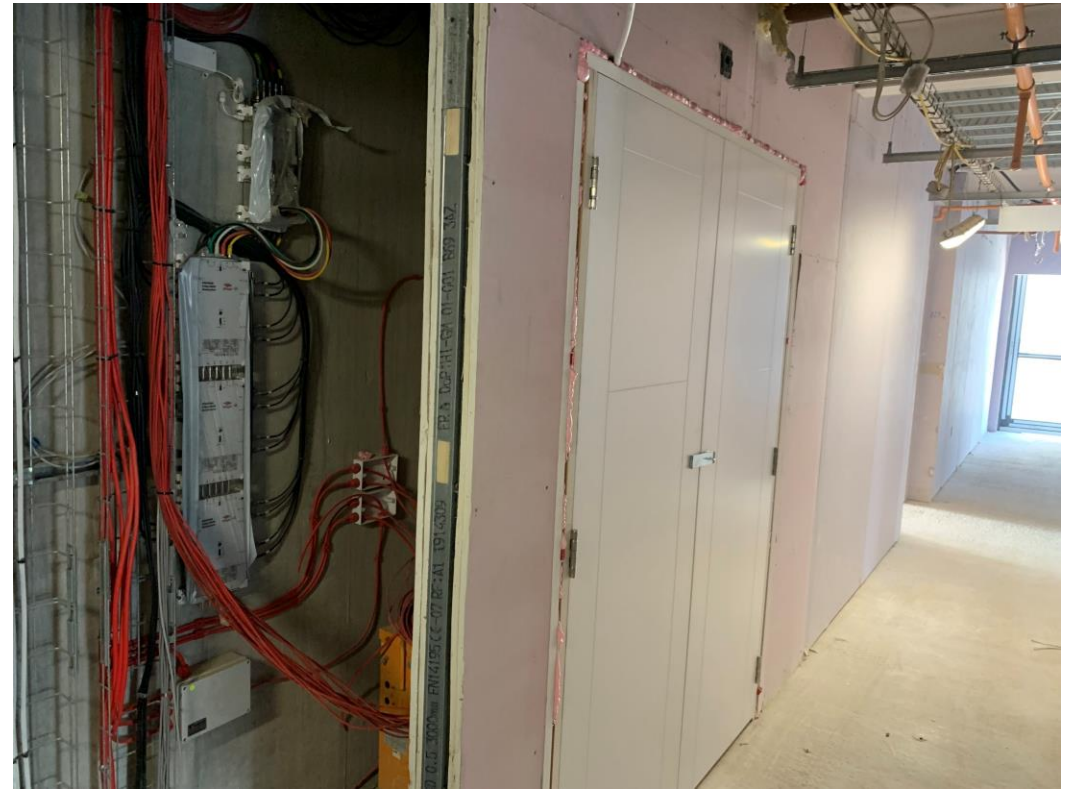
Temporary fire doors installed to services cupboard
