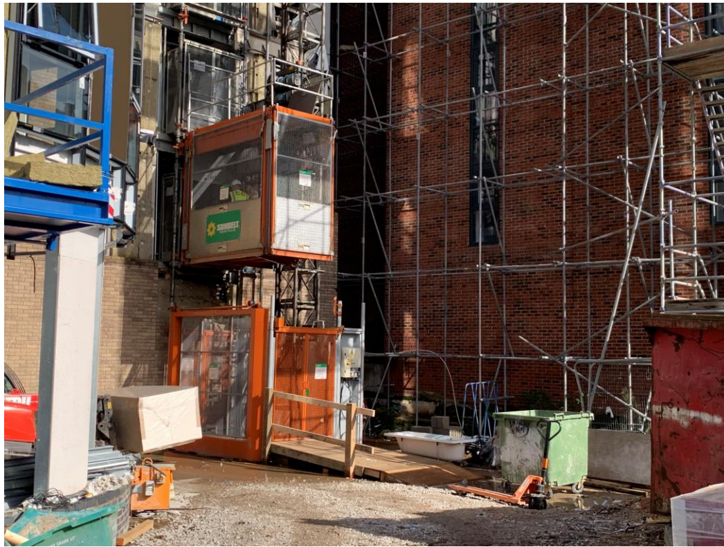
Hoist lift installation complete
