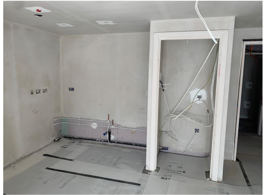
Kitchen 1 st fix plumbing and electrics. Boiler door removed
