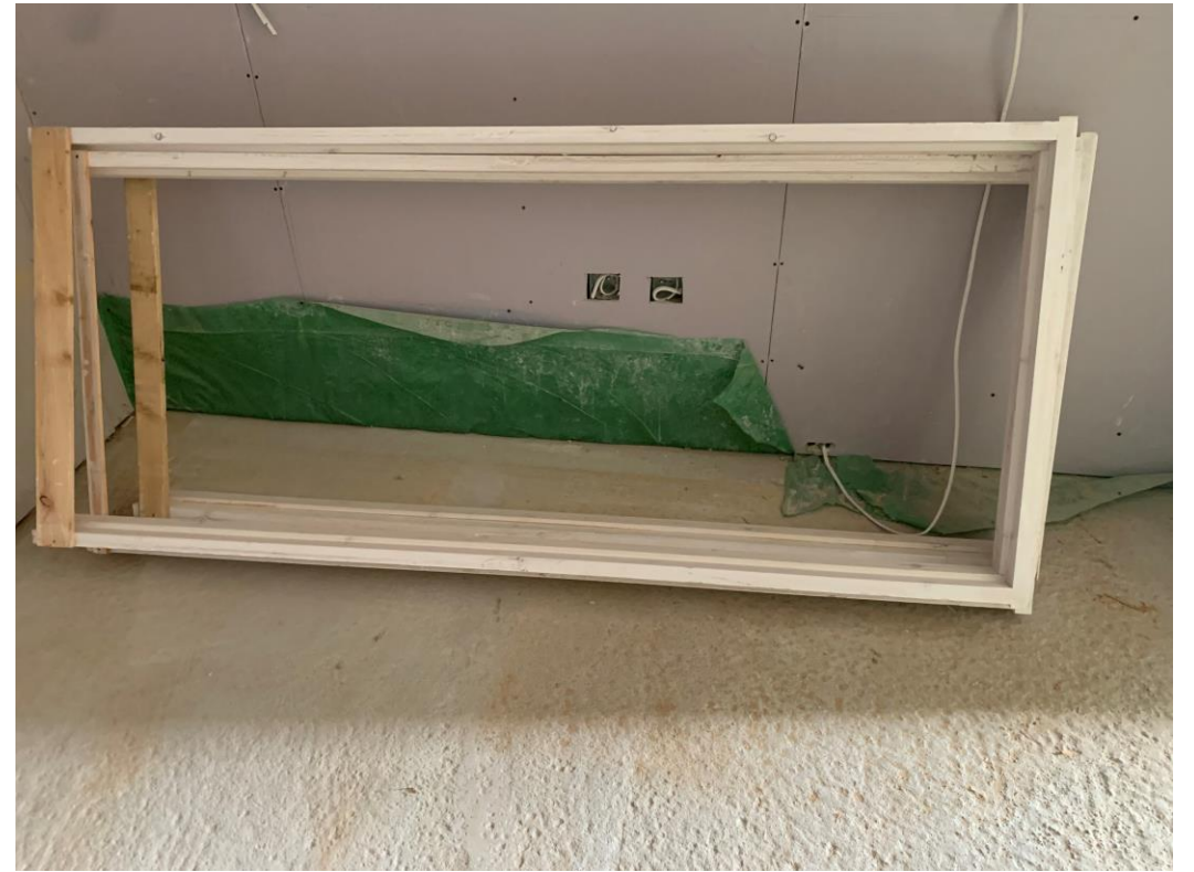
New door frames ready to be installed
