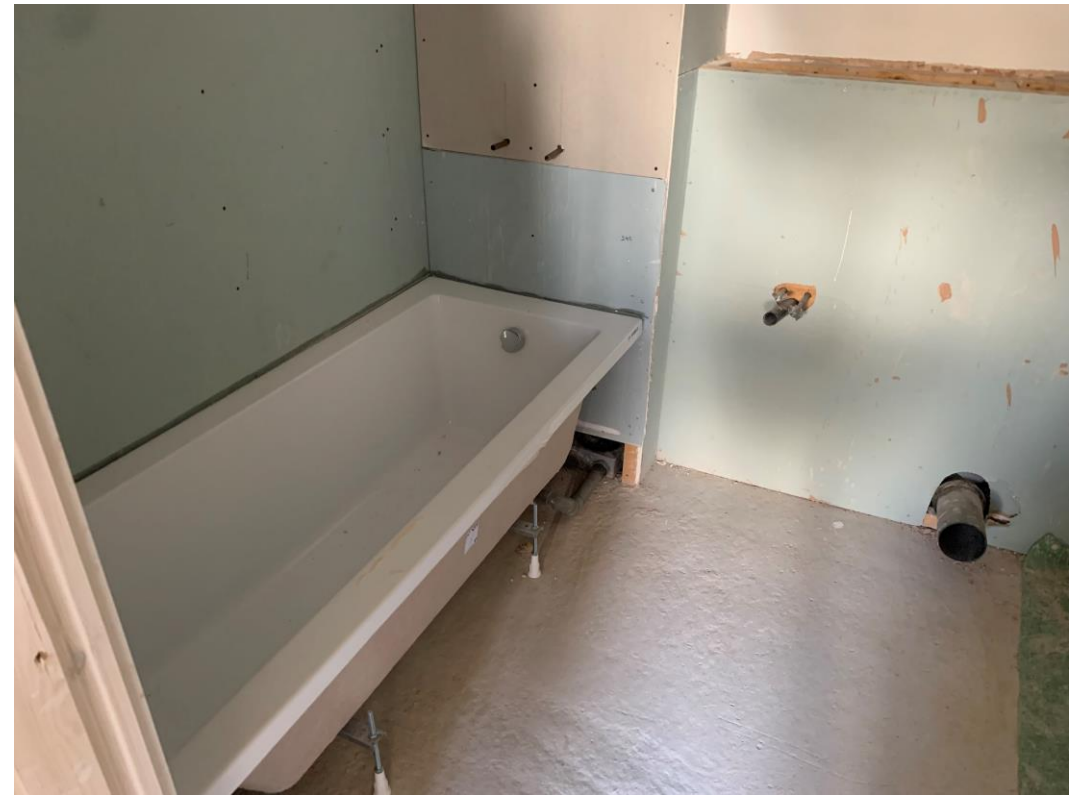
New bathroom sanitary fittings installation ongoing
