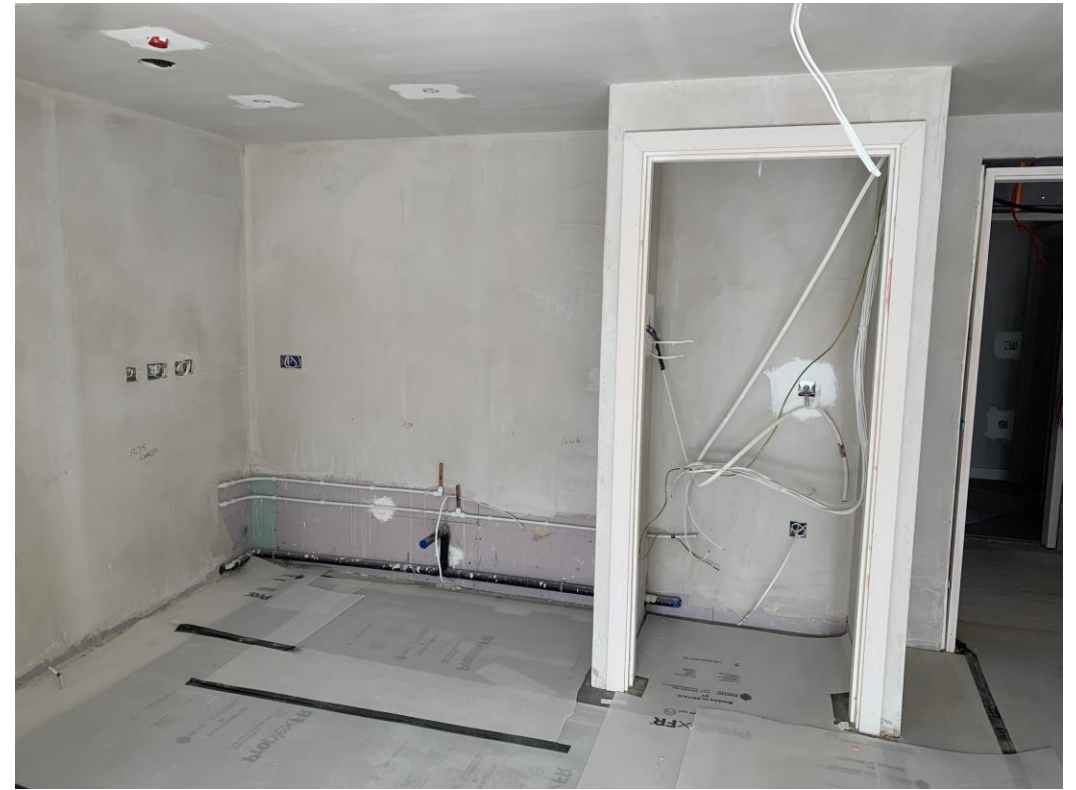
Kitchen removal complete
