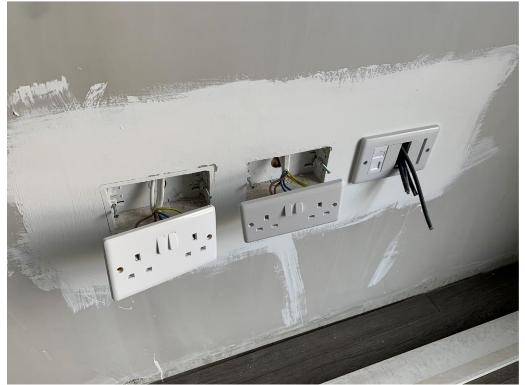
New 2 nd fix electrics
