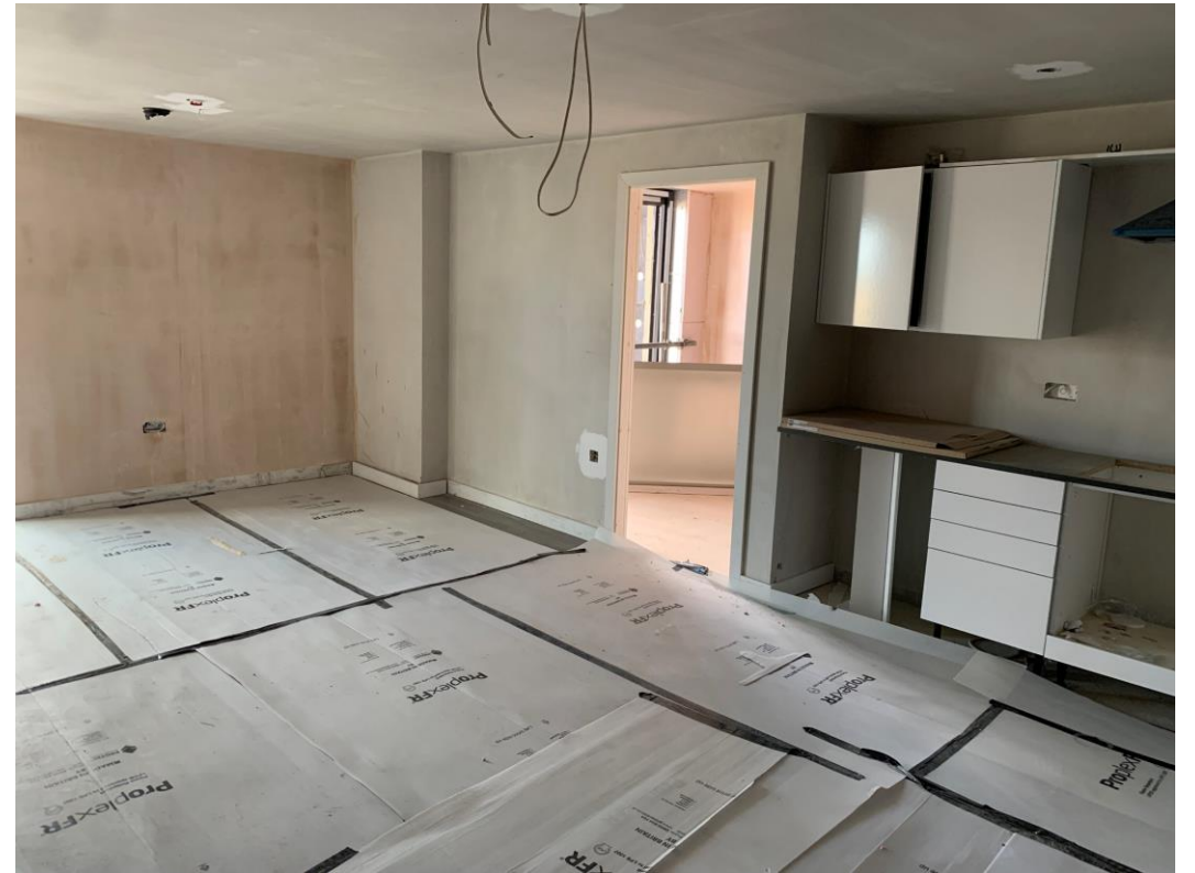
Floor finishes installed & protected
