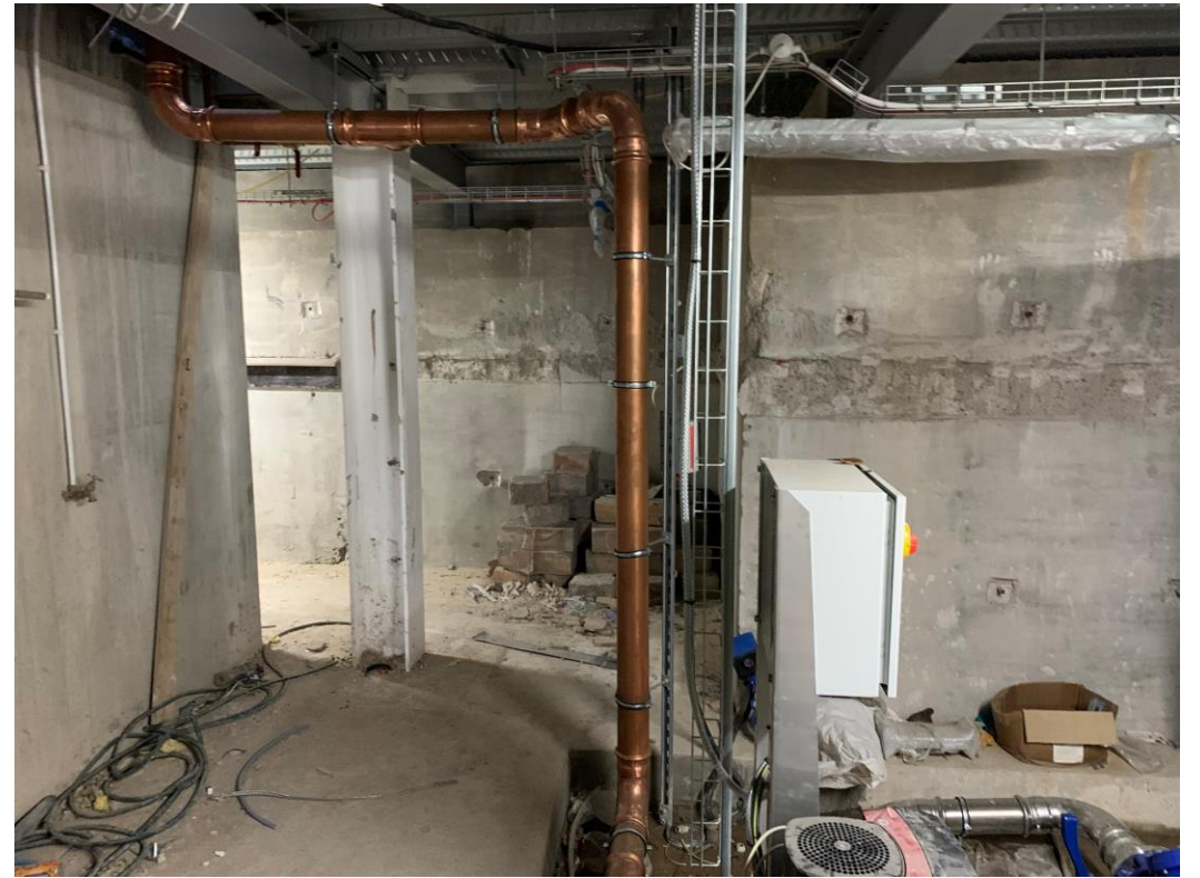
Electrical services installation ongoing
