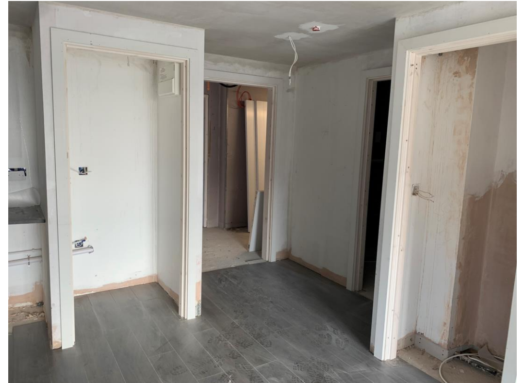
All doors removed throughout all apartment
