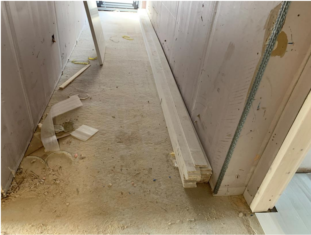
New skirting boards ready to be installed
