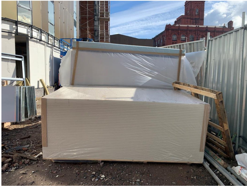
Site material storage
