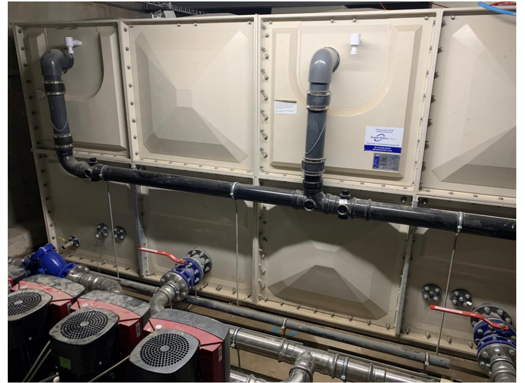
Basement Plant room fit out ongoing
