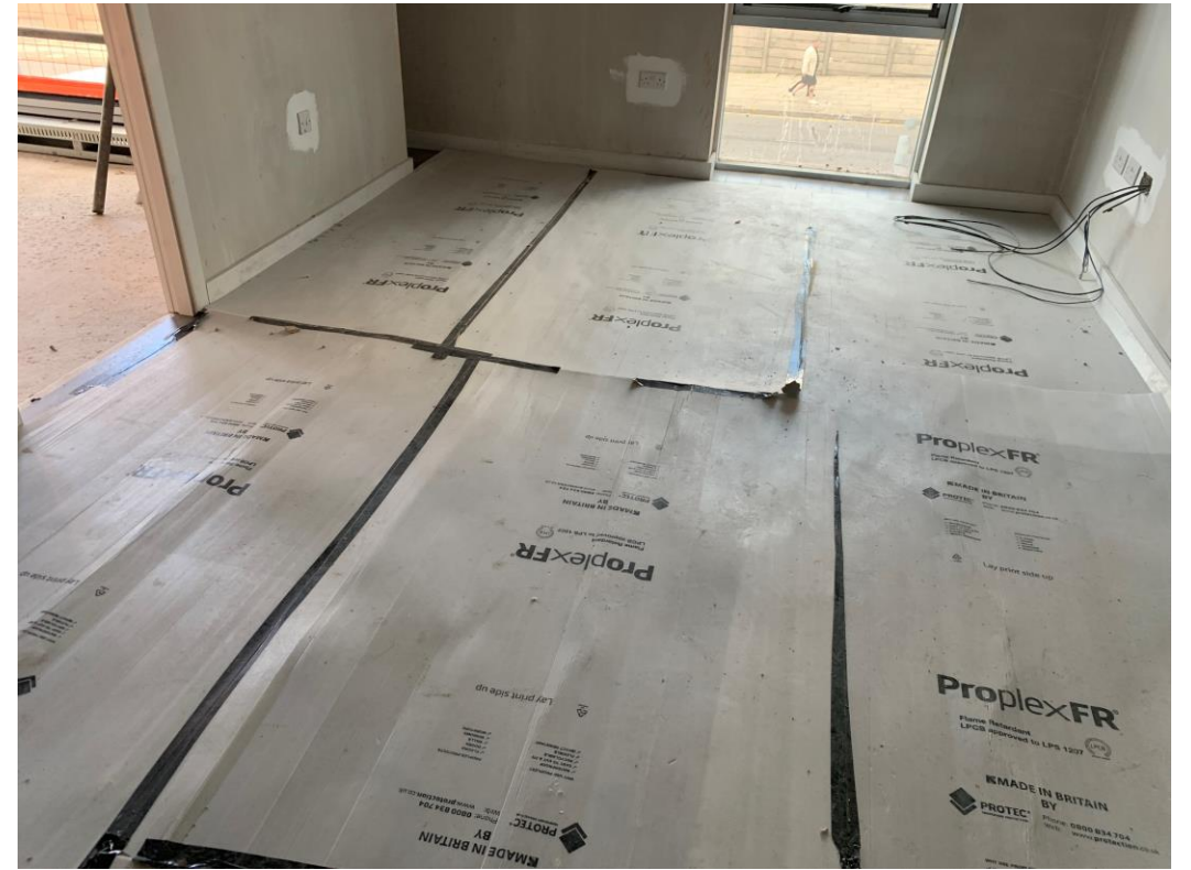
Floor finishes installed & protected
