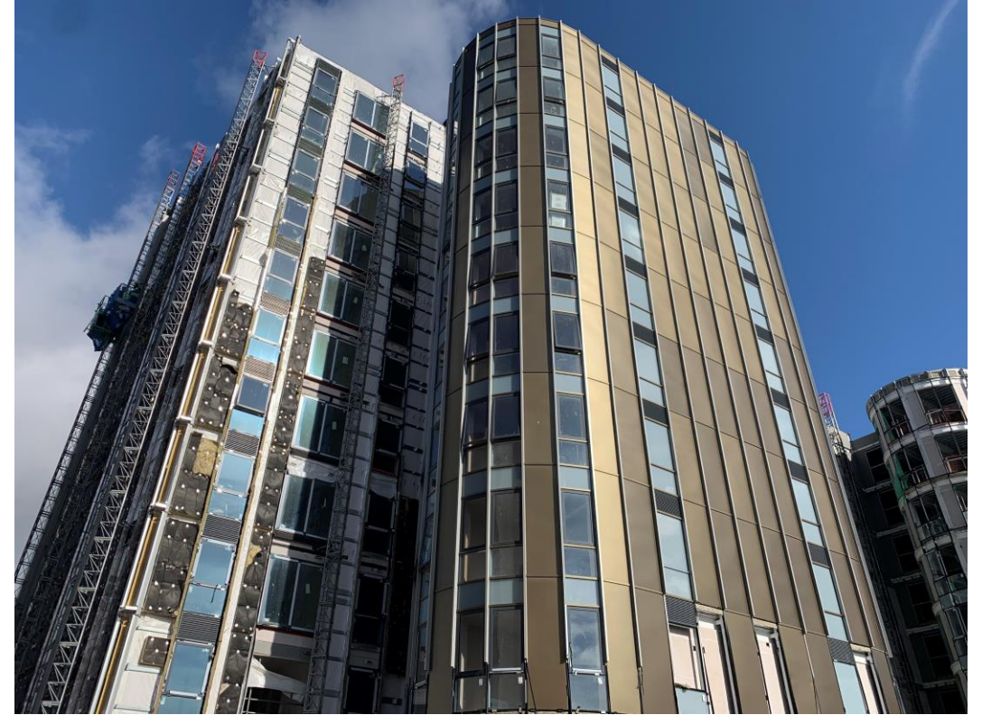
Development viewed from Caryl street
