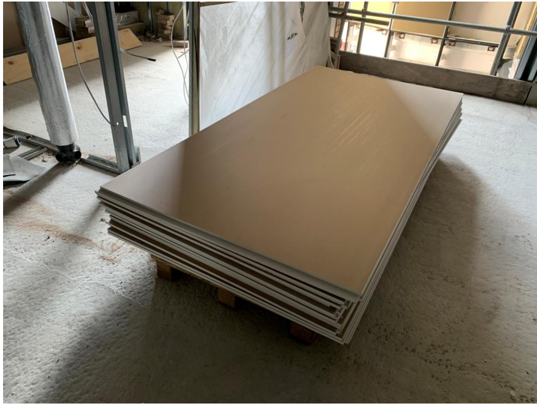
On-site material storage
