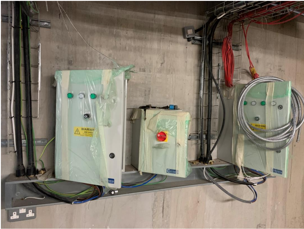
Electrical services installation ongoing
