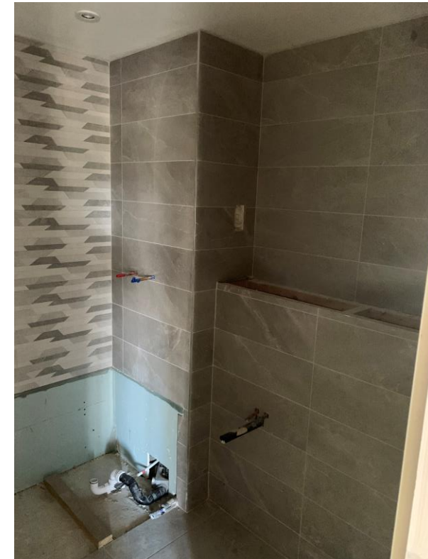
Sample wall tiling for the new bathroom suite
