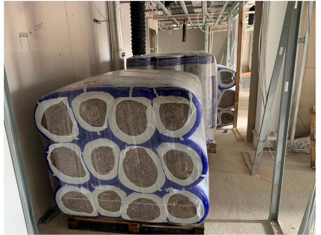
Cladding insulation storage
