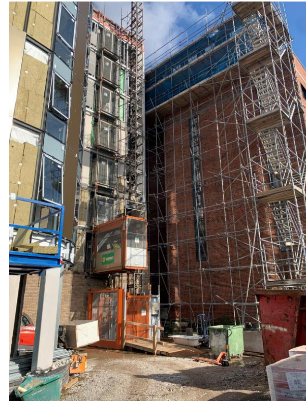
Hoist lift installation complete
