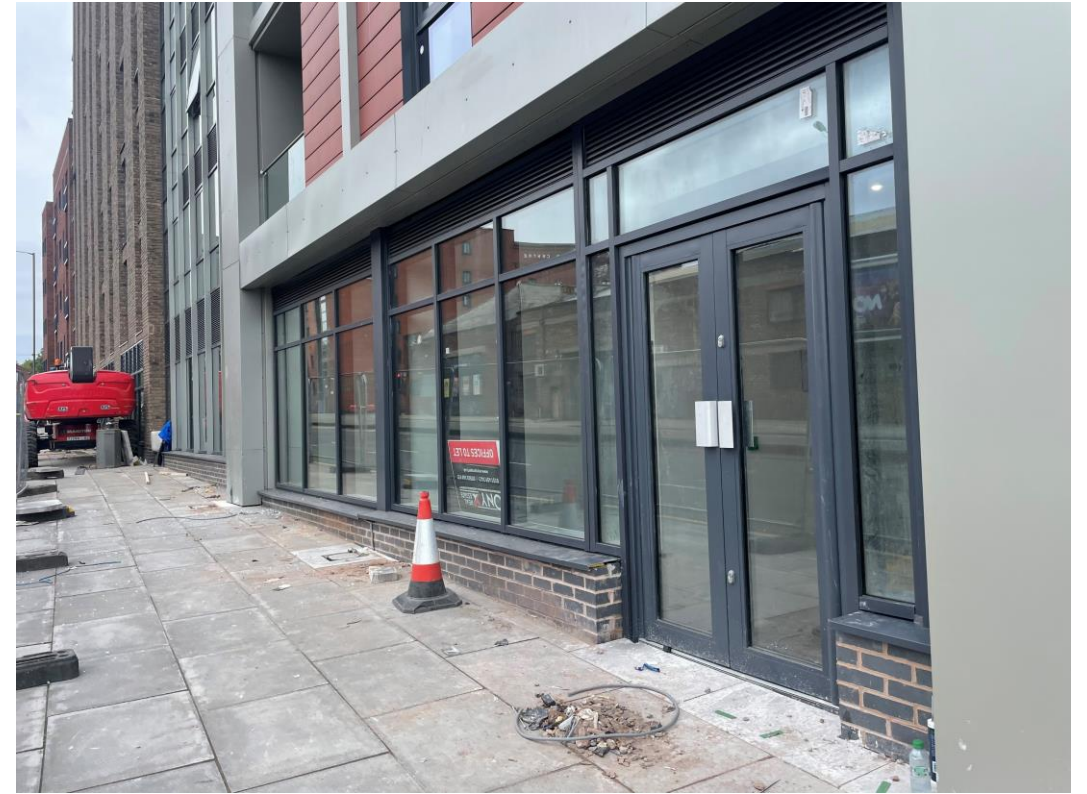
Curtain walling, windows & doors installed
