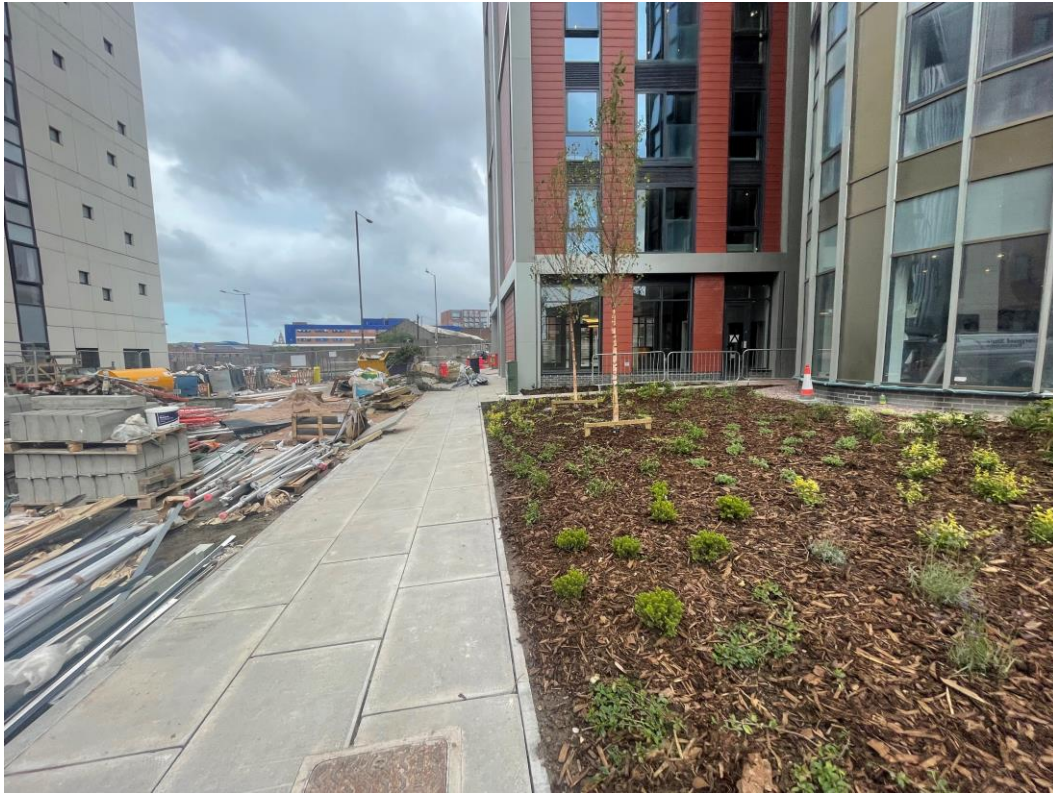
Landscaping works ongoing to Caryl Street elevations
