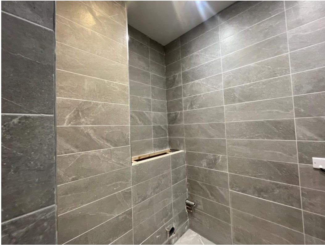
Bathroom walls tiled
