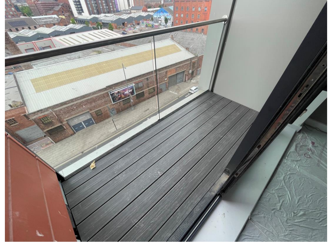
Glazed balustrade installed
