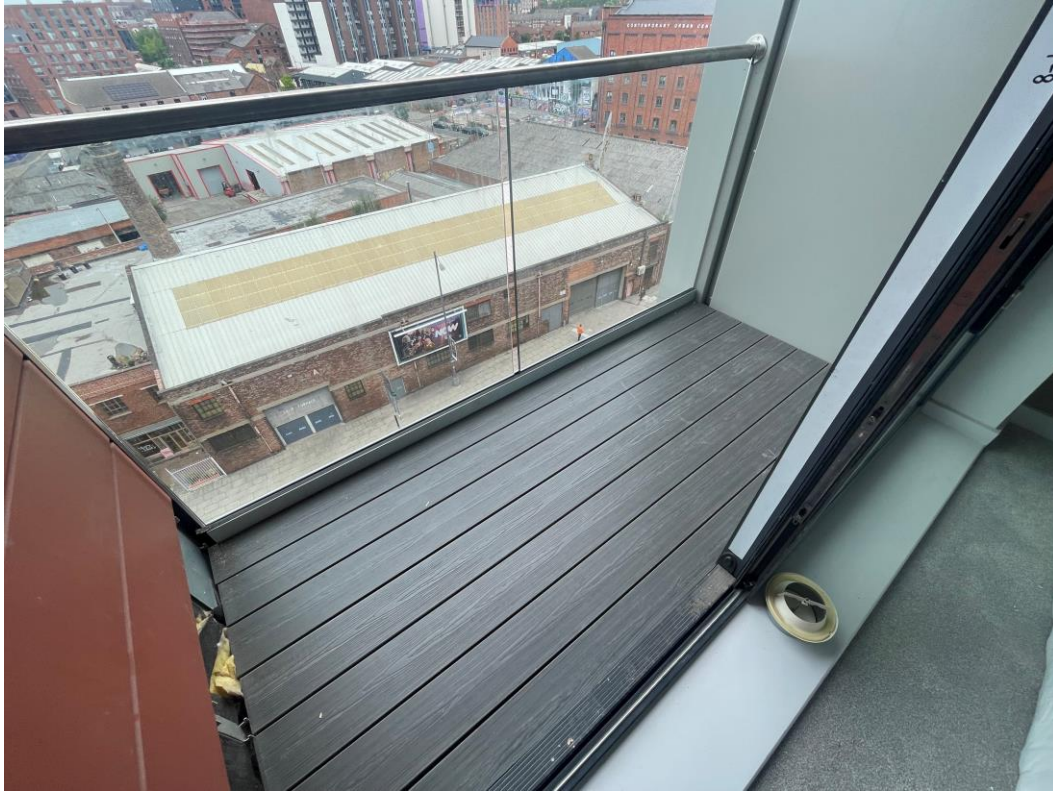
Balcony composite decking installed
