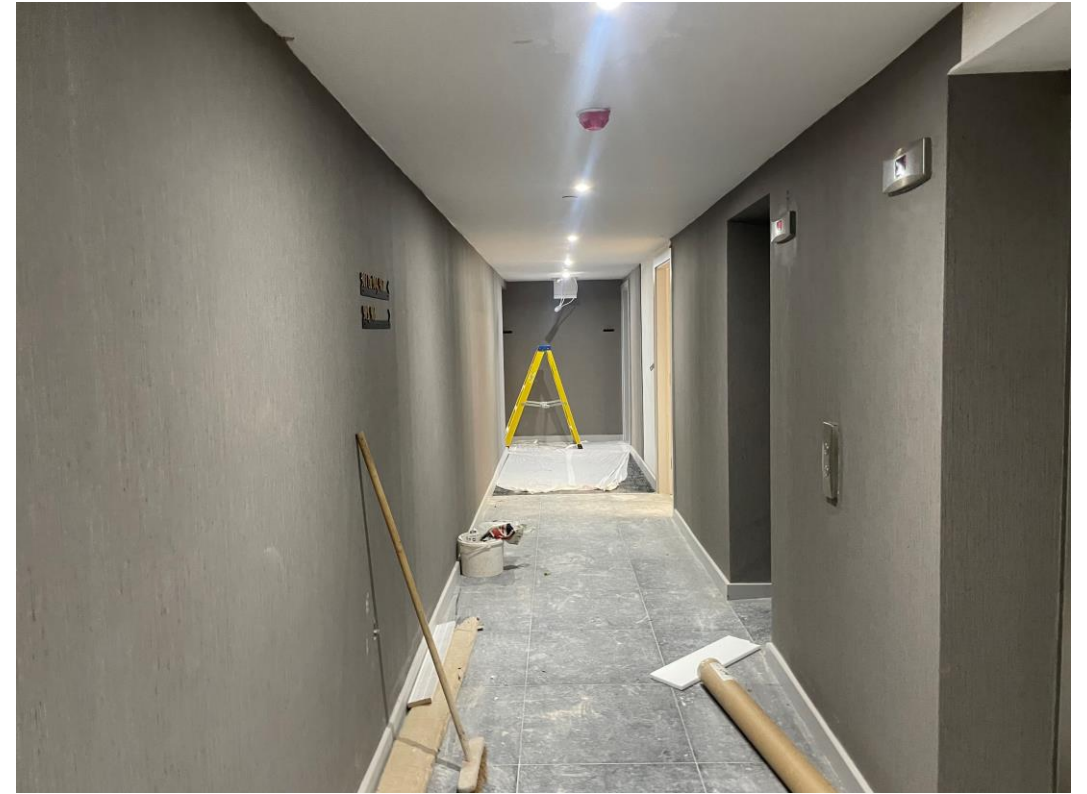
Circulation area finishes
