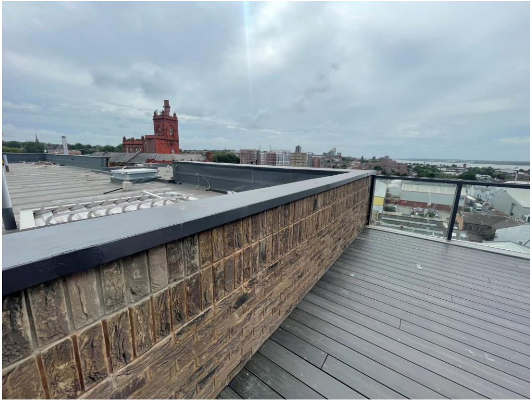
Parapet capping's installed
