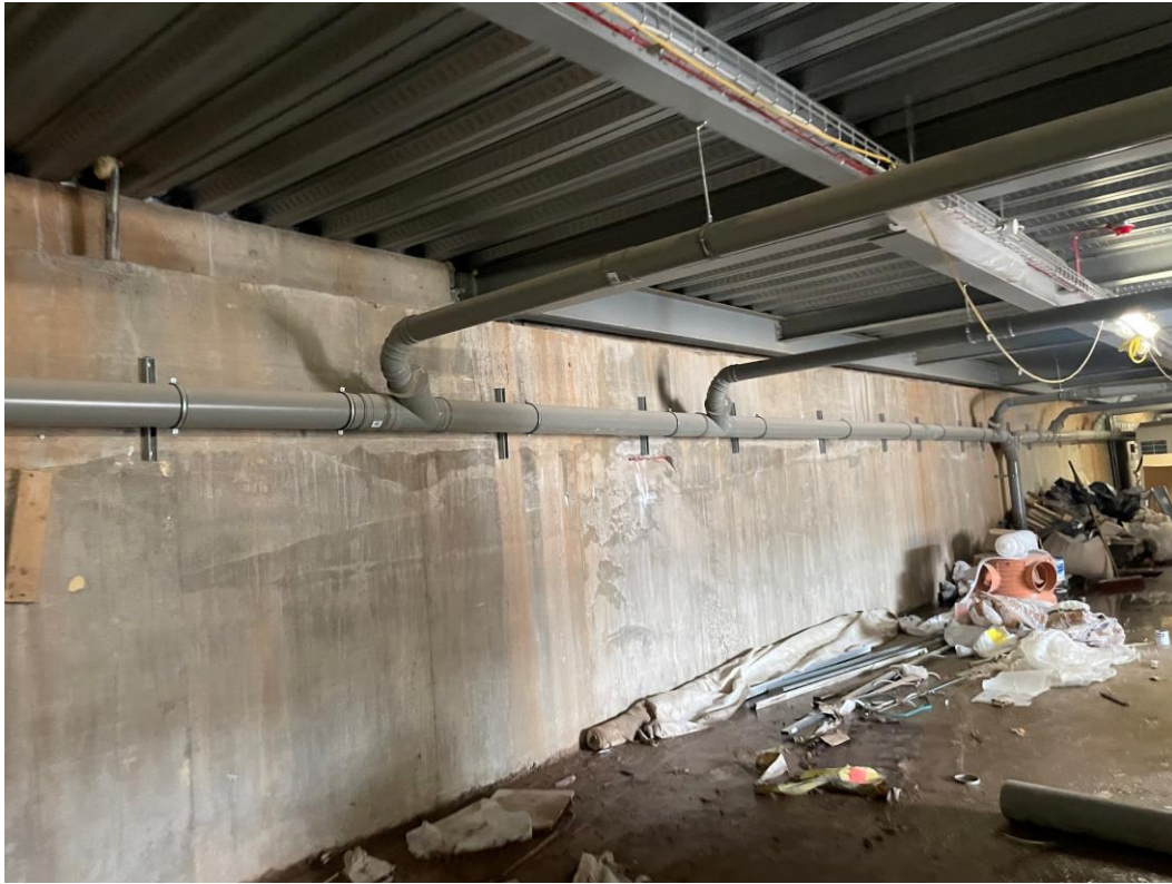
Above ground drainage installation ongoing
