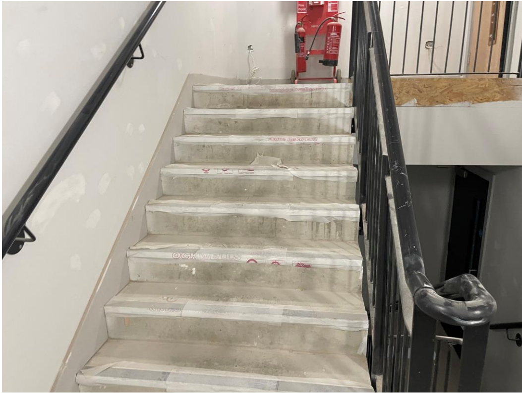
Stair nosing installed
