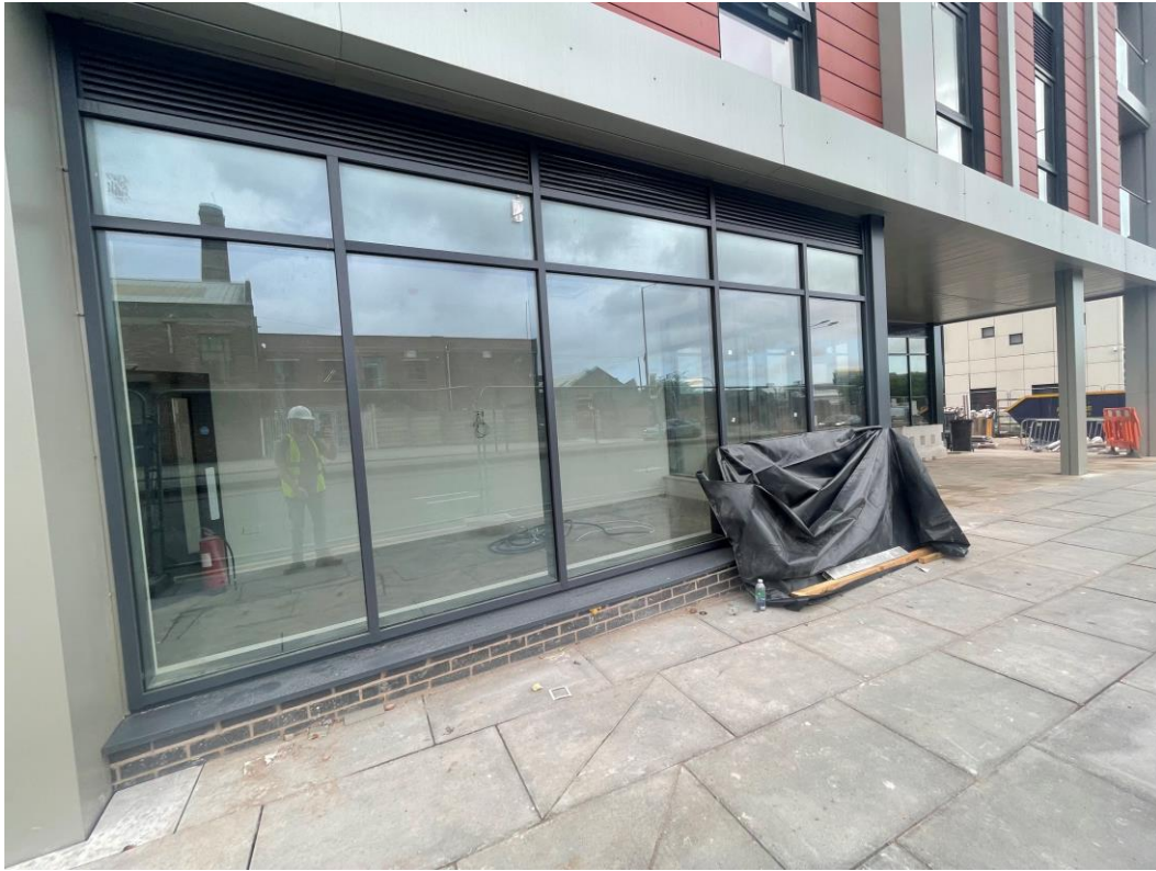
Curtain walling, windows & doors installed
