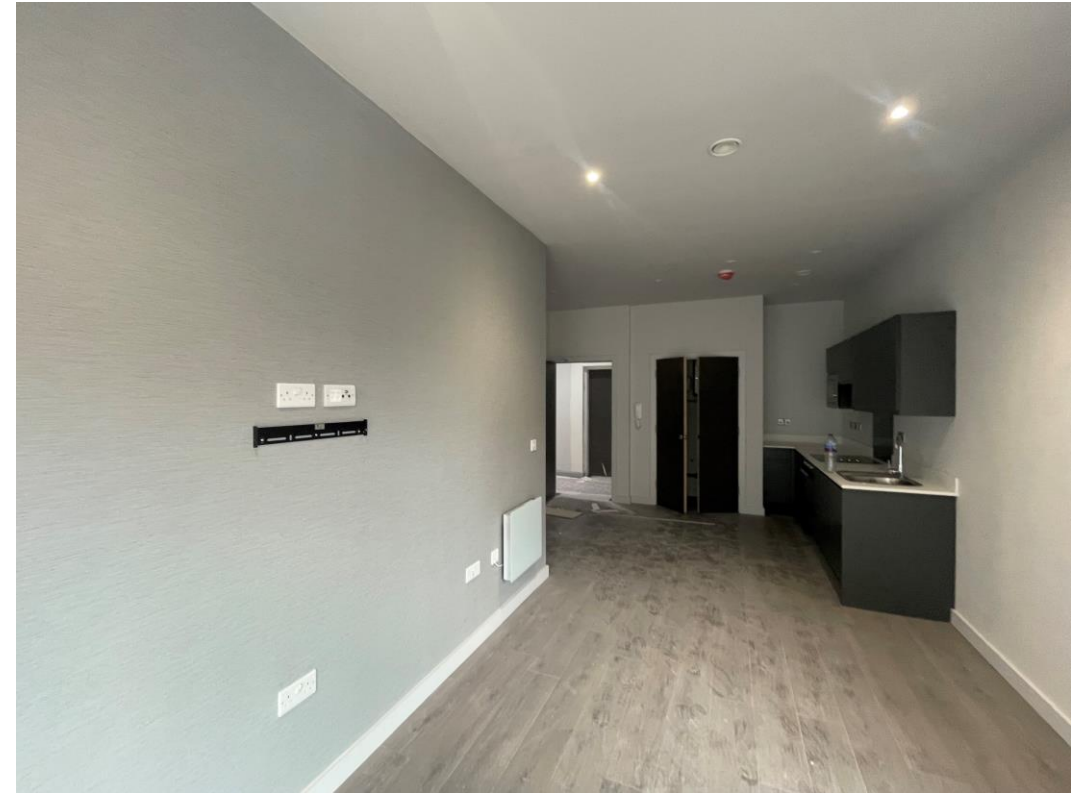
Kitchen / Lounge finishes
