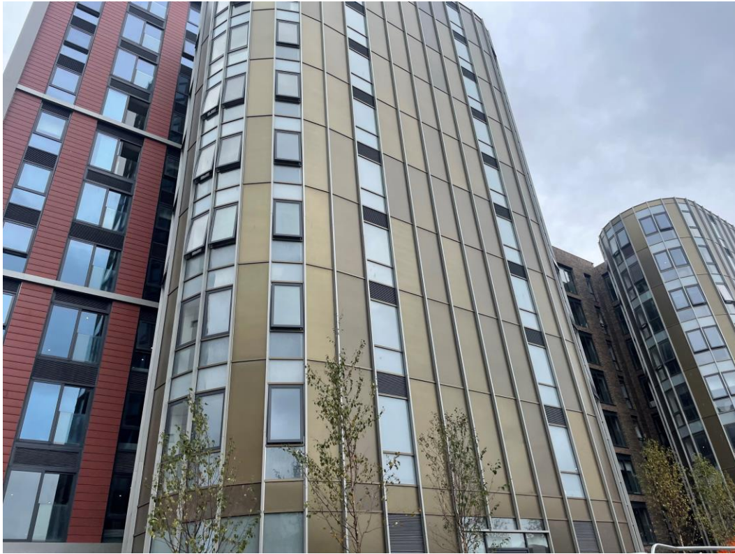
Brindley Street site view
