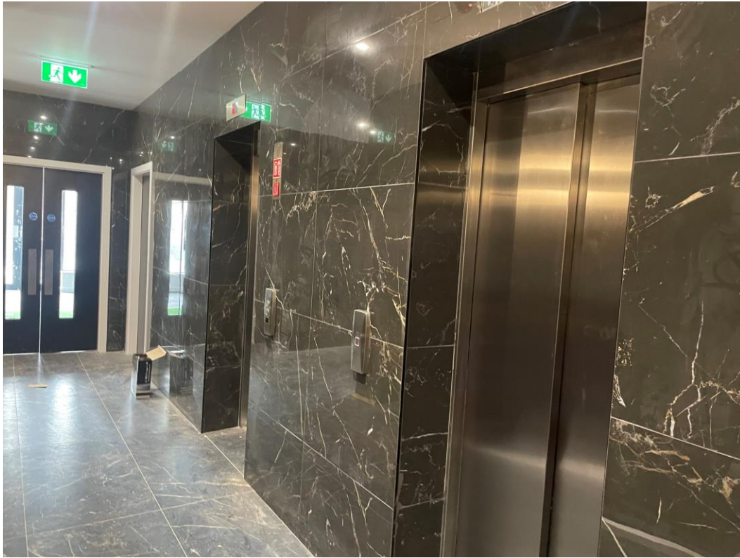
Lift lobby finishes
