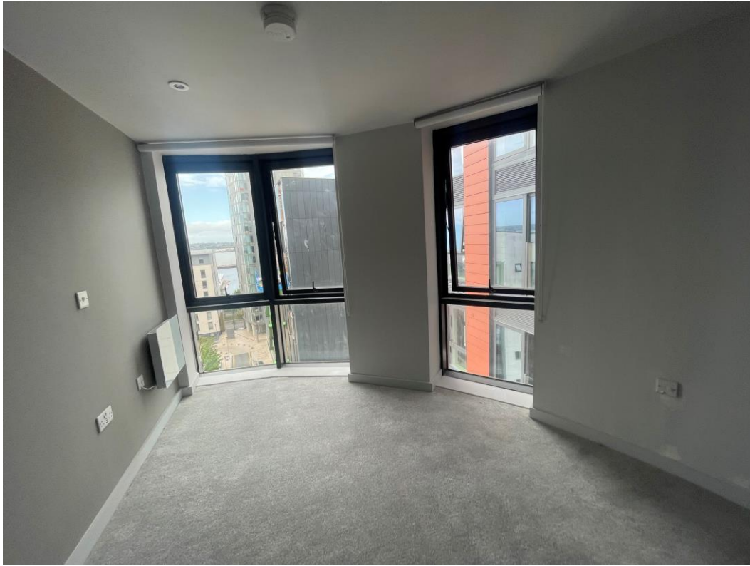
Bedroom finishes ongoing
