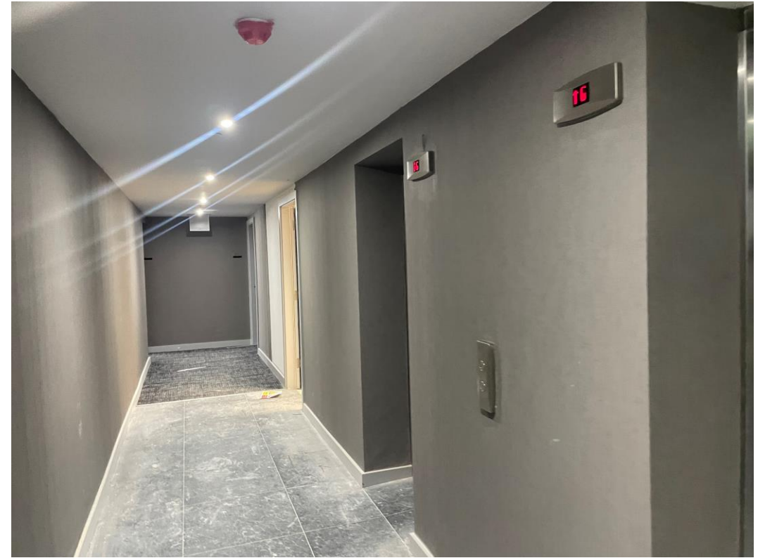
Circulation area finishes
