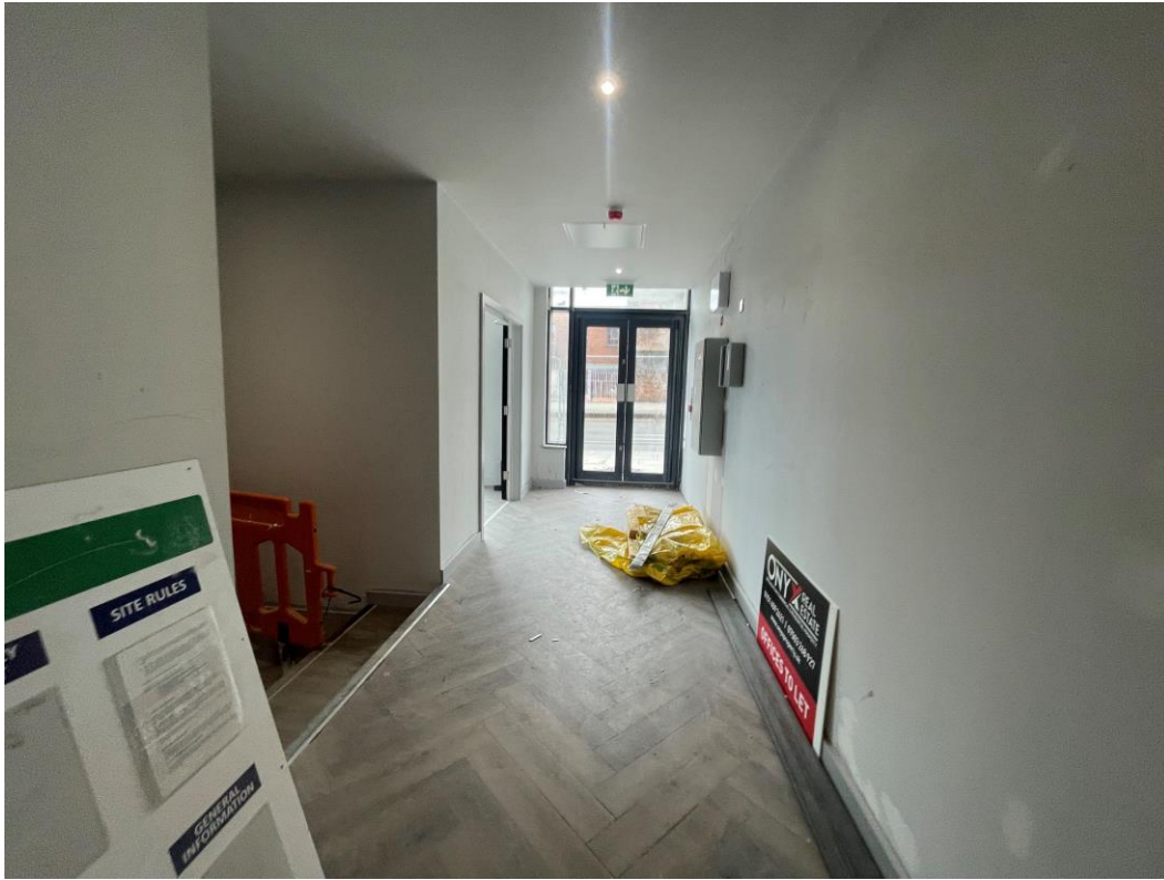
Circulation area finishes ongoing
