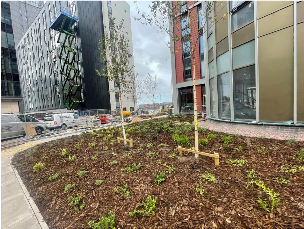
Landscaping works ongoing to Brindley Street elevations
