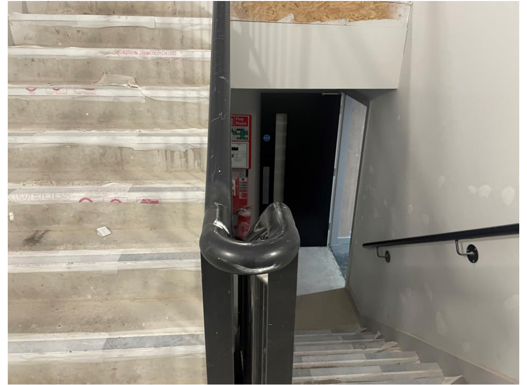
Handrail finishes ongoing
