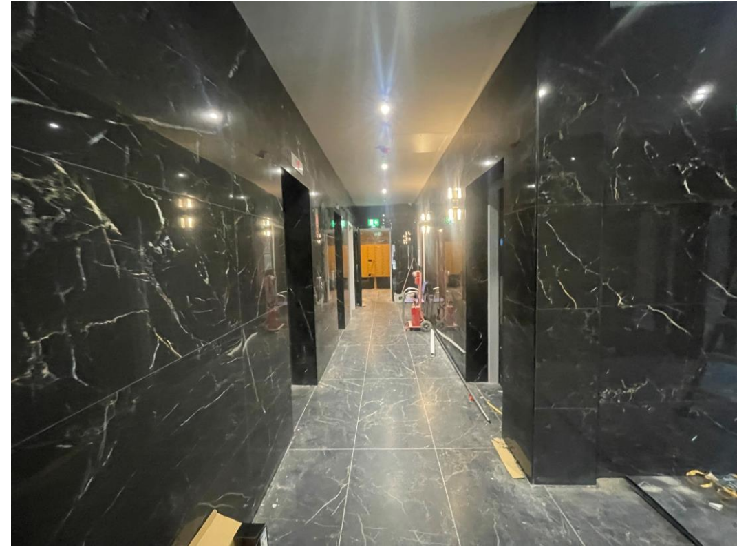
Lift lobby finishes
