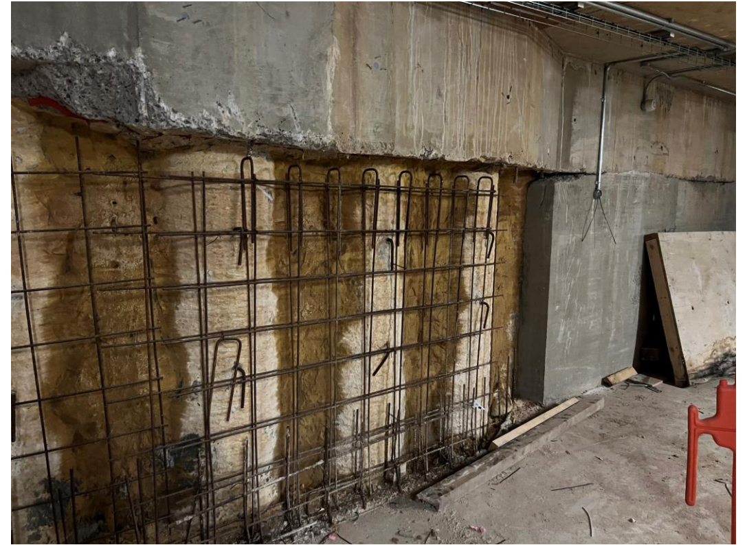
Concrete infill ongoing to basement area
