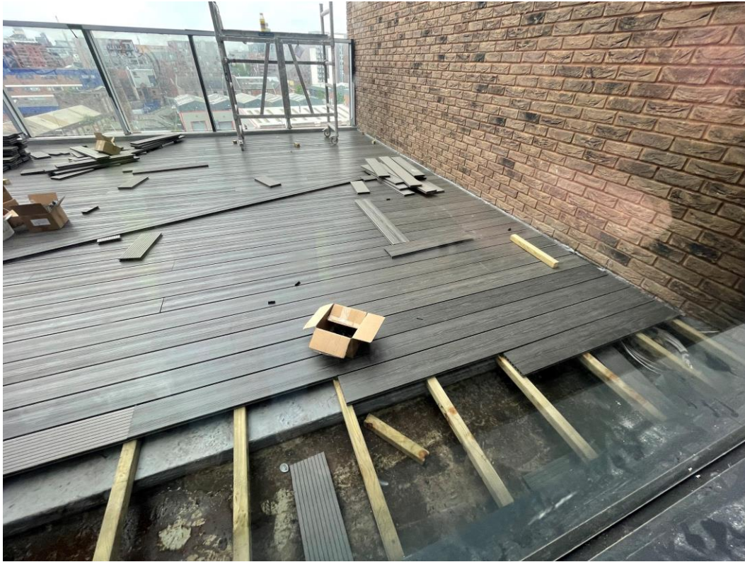
Composite decking installation
