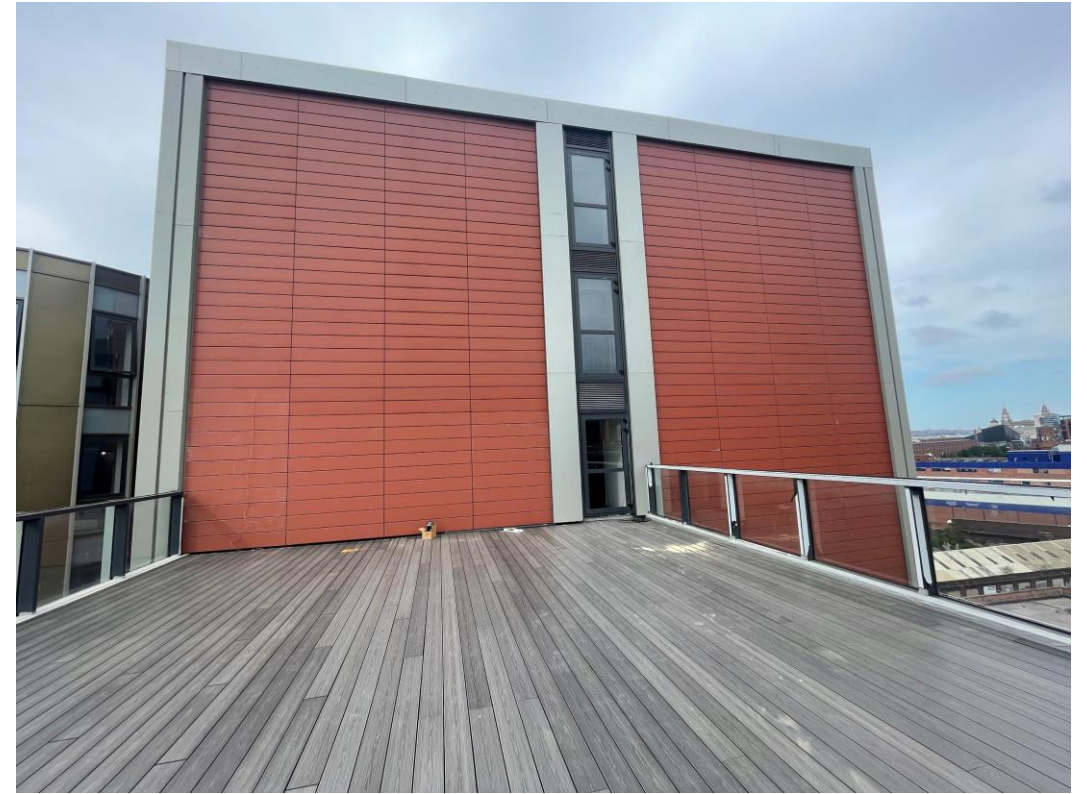
Composite decking installed
