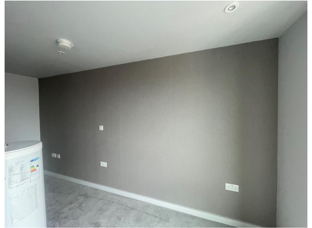
Feature wall installed to bedrooms
