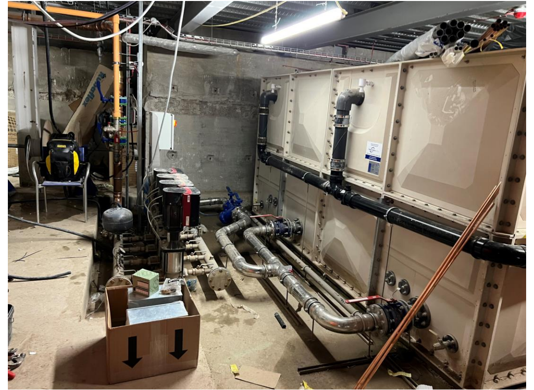
Water tank & pump installation complete
