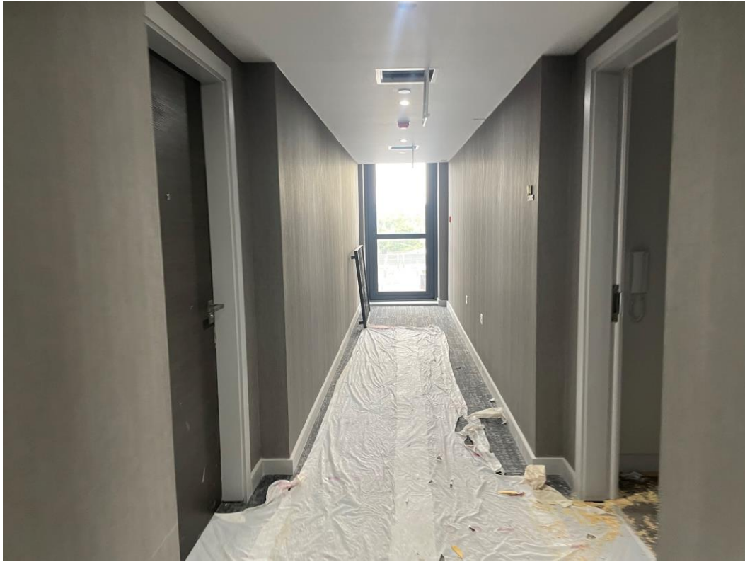
Circulation area finishes
