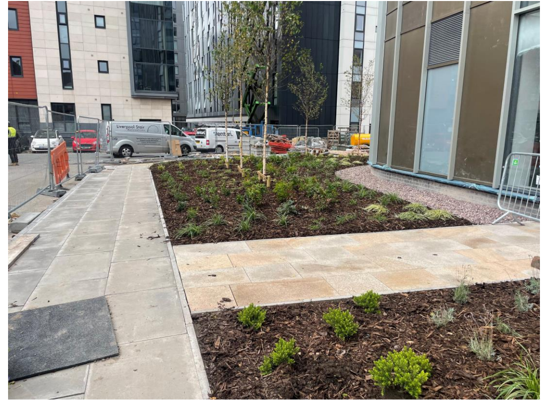
Landscaping works ongoing to Brindley Street elevations
