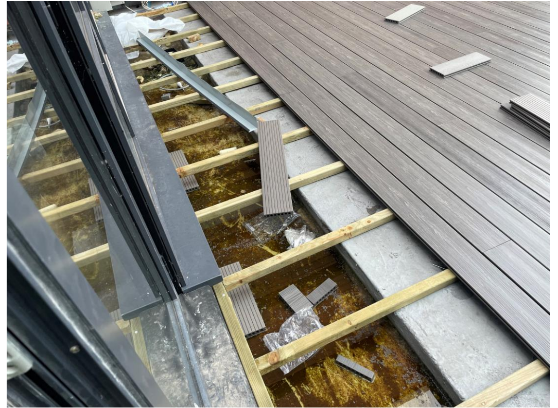
Composite decking installation
