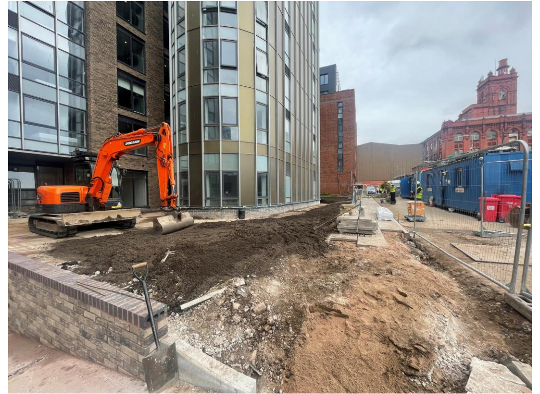
Landscaping works ongoing to Brindley Street elevations
