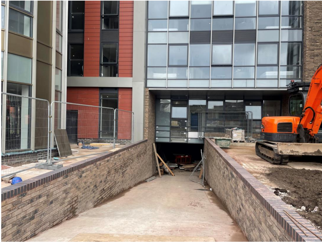
Brickwork complete to basement ramp
