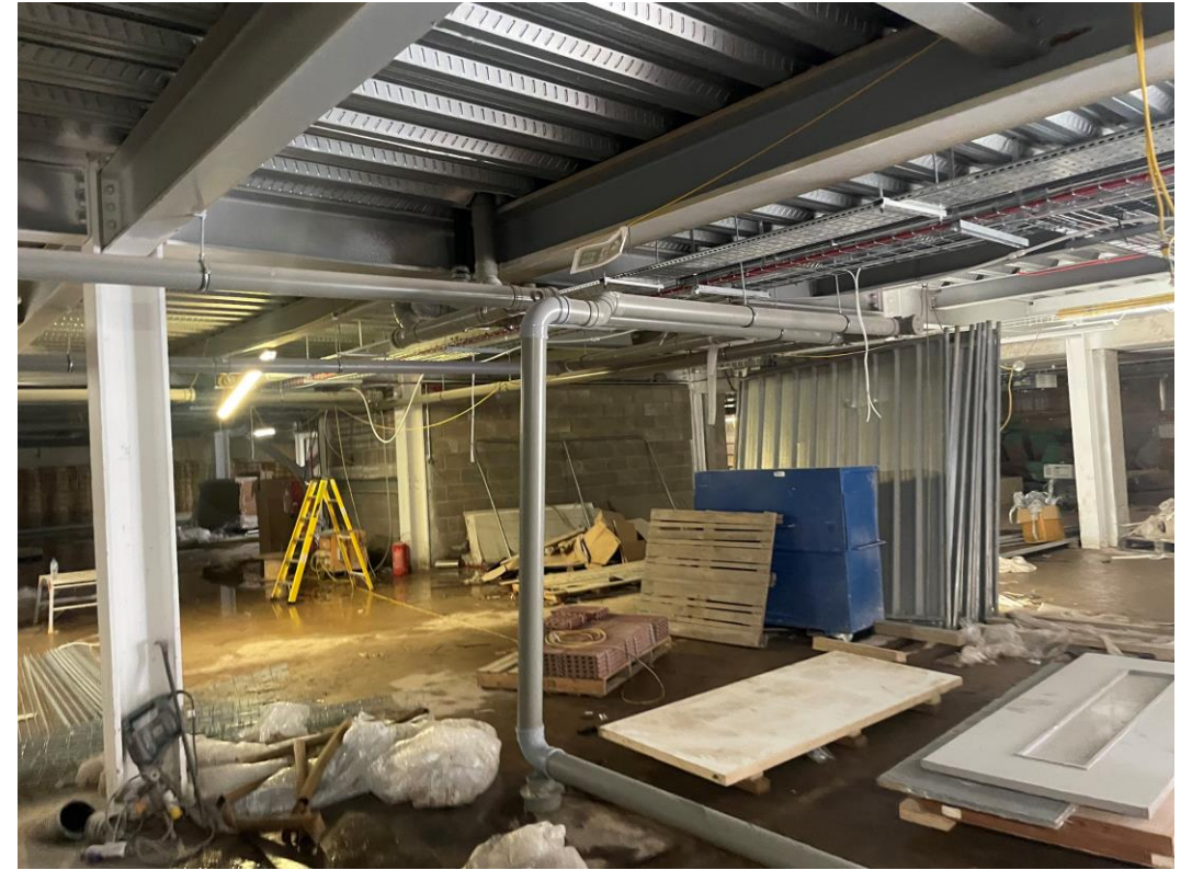
Above ground drainage installation ongoing
