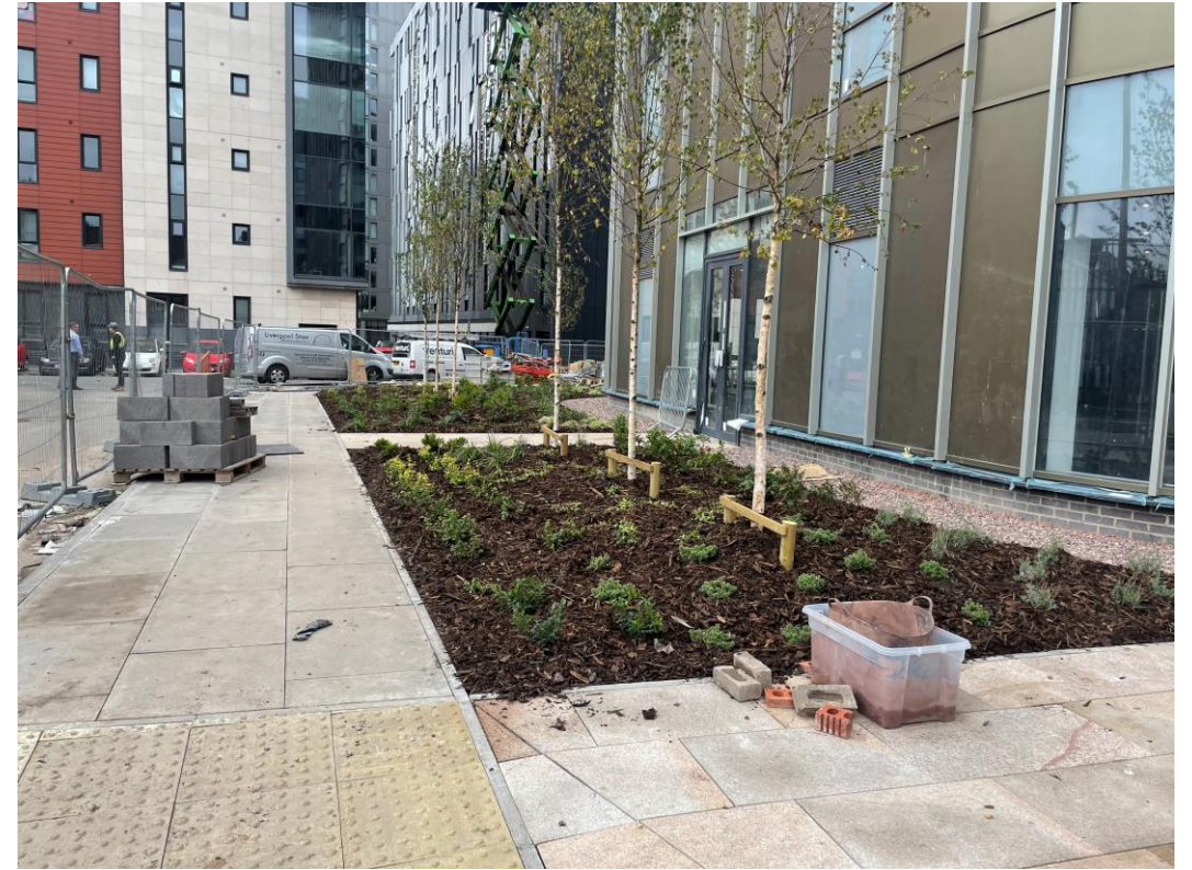
Landscaping works ongoing to Brindley Street elevations
