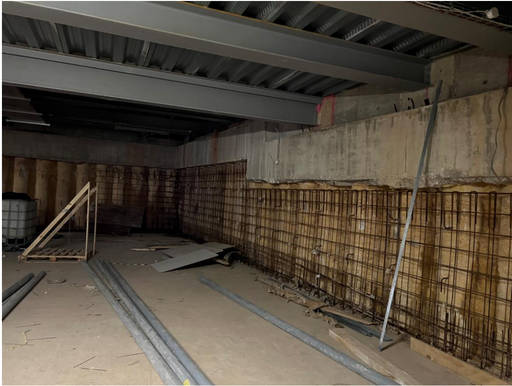
Concrete infill ongoing to basement area
