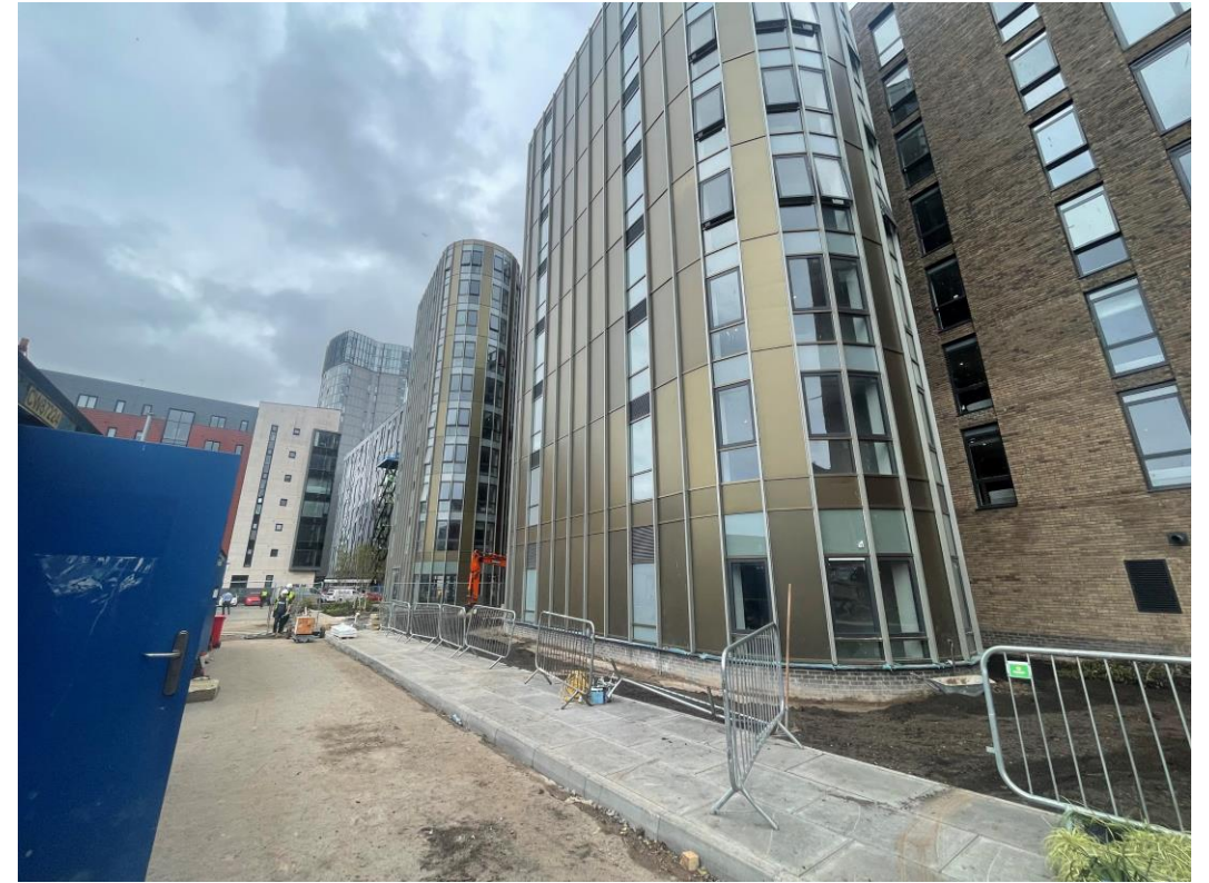
Landscaping works ongoing to Brindley Street elevations
