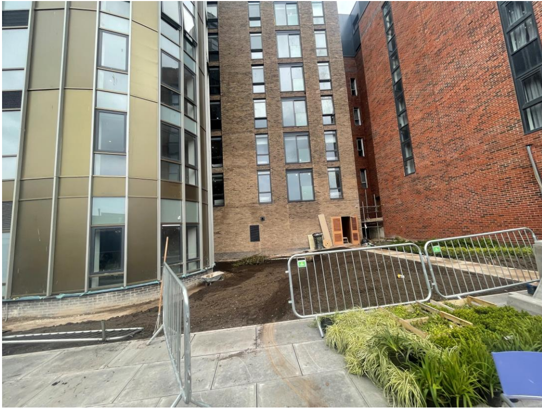
Landscaping works ongoing to Brindley Street elevations
