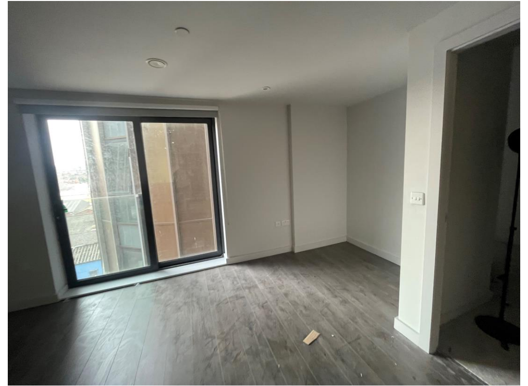
Lounge finishes ongoing
