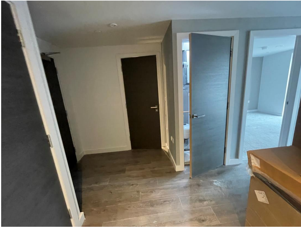
Apartment doors & ironmongery installed
