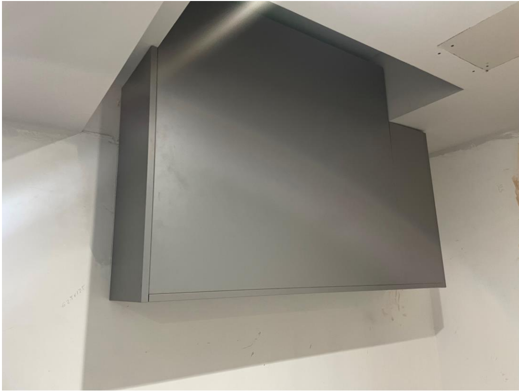
Power isolation for lift boxed in
