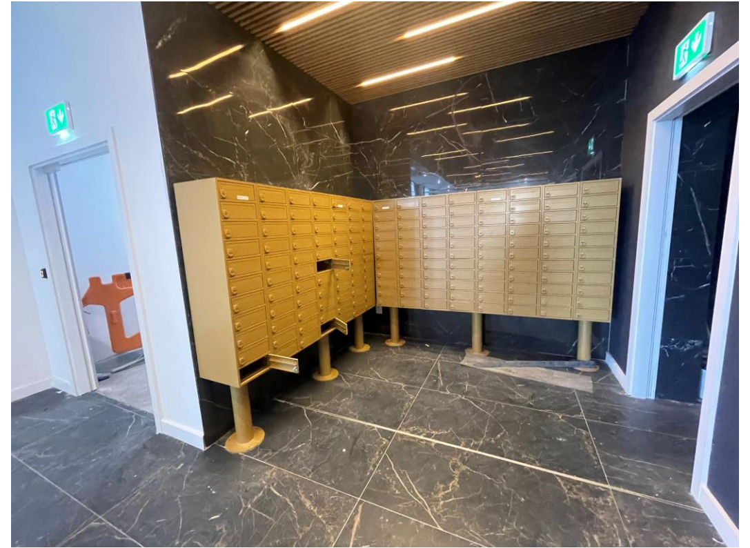
Letter boxes installed
