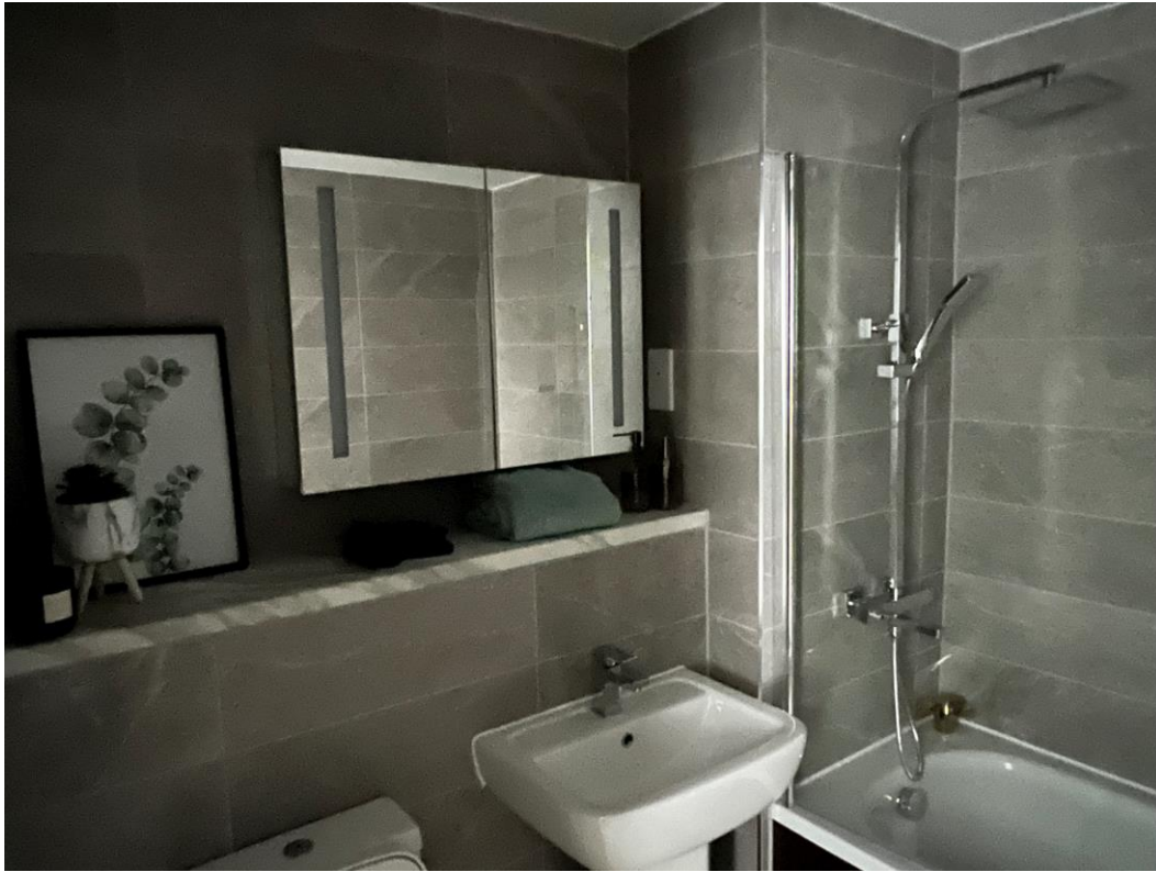
Show Flat – Bathroom Sanitary Items
