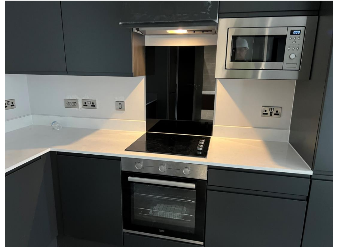
Kitchen appliances installed
