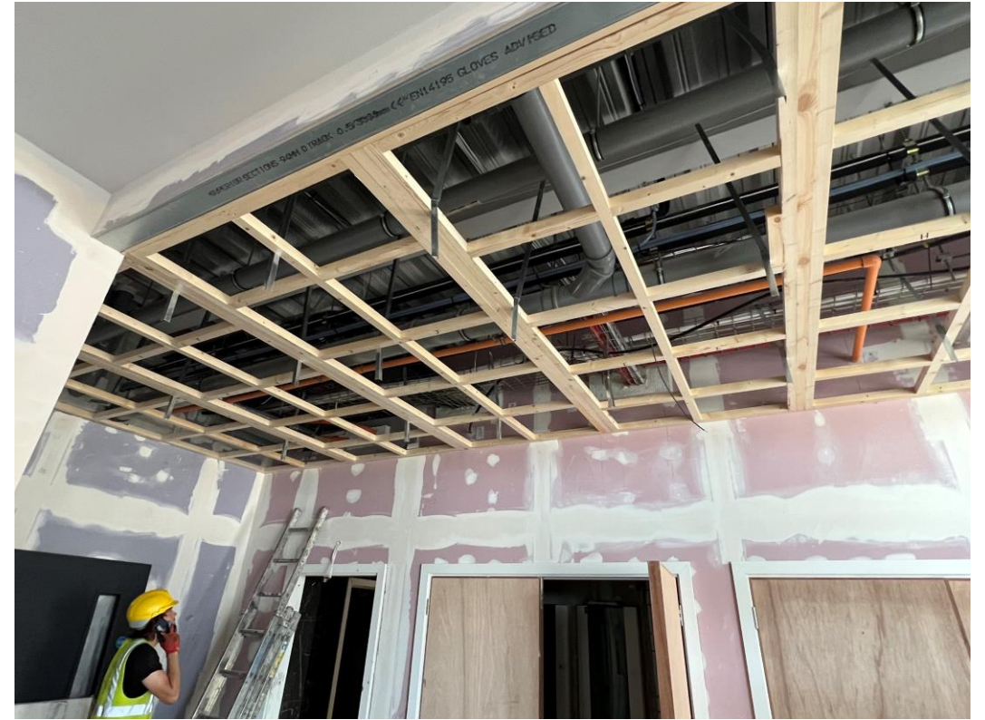
Ground Floor – Reception desk ceiling framework
