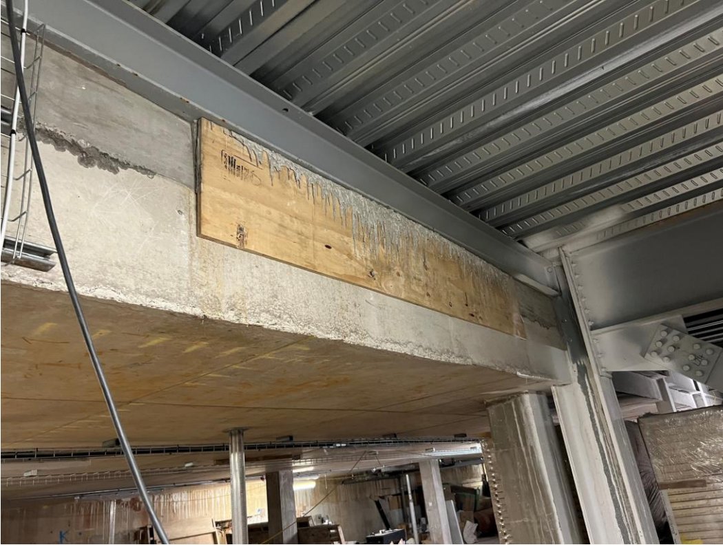
Shuttering installed for concrete infill
