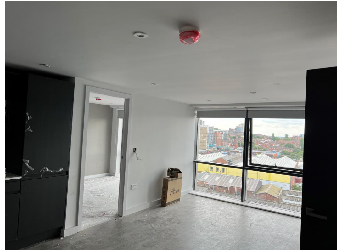
Lounge finishes ongoing
