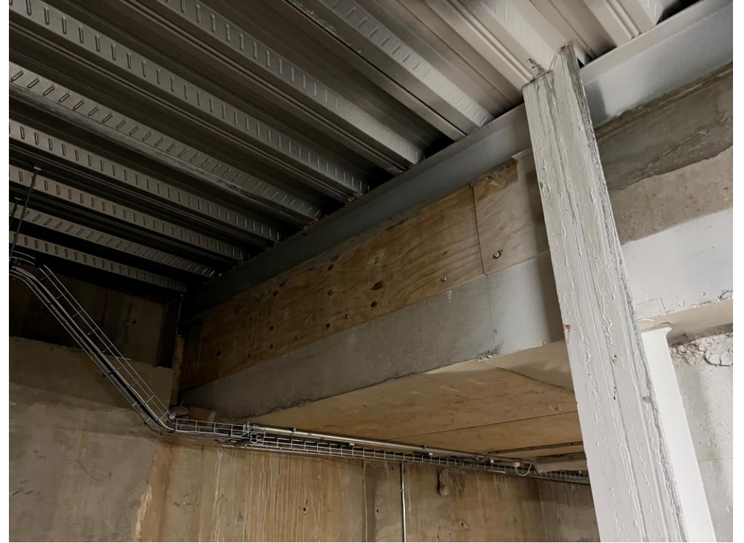
Concrete infill ongoing to basement area
