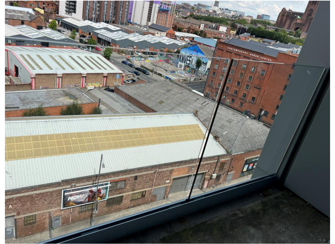
Glazed balustrade installed
