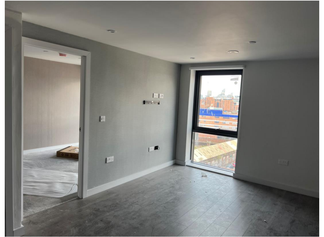
Feature wall installation to lounge
