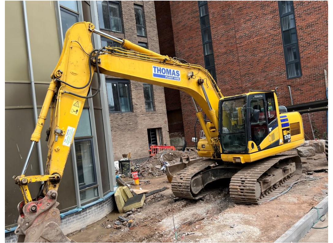
Plant in use onsite
