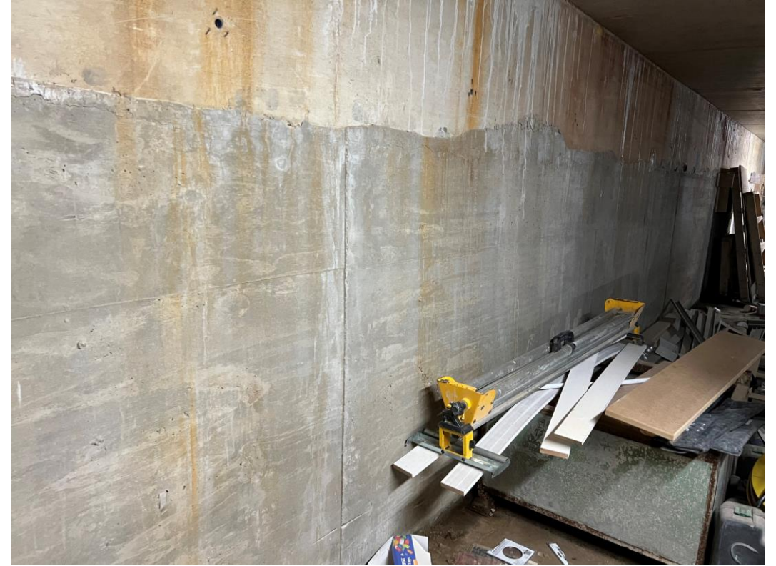
Concrete infill ongoing to basement area
