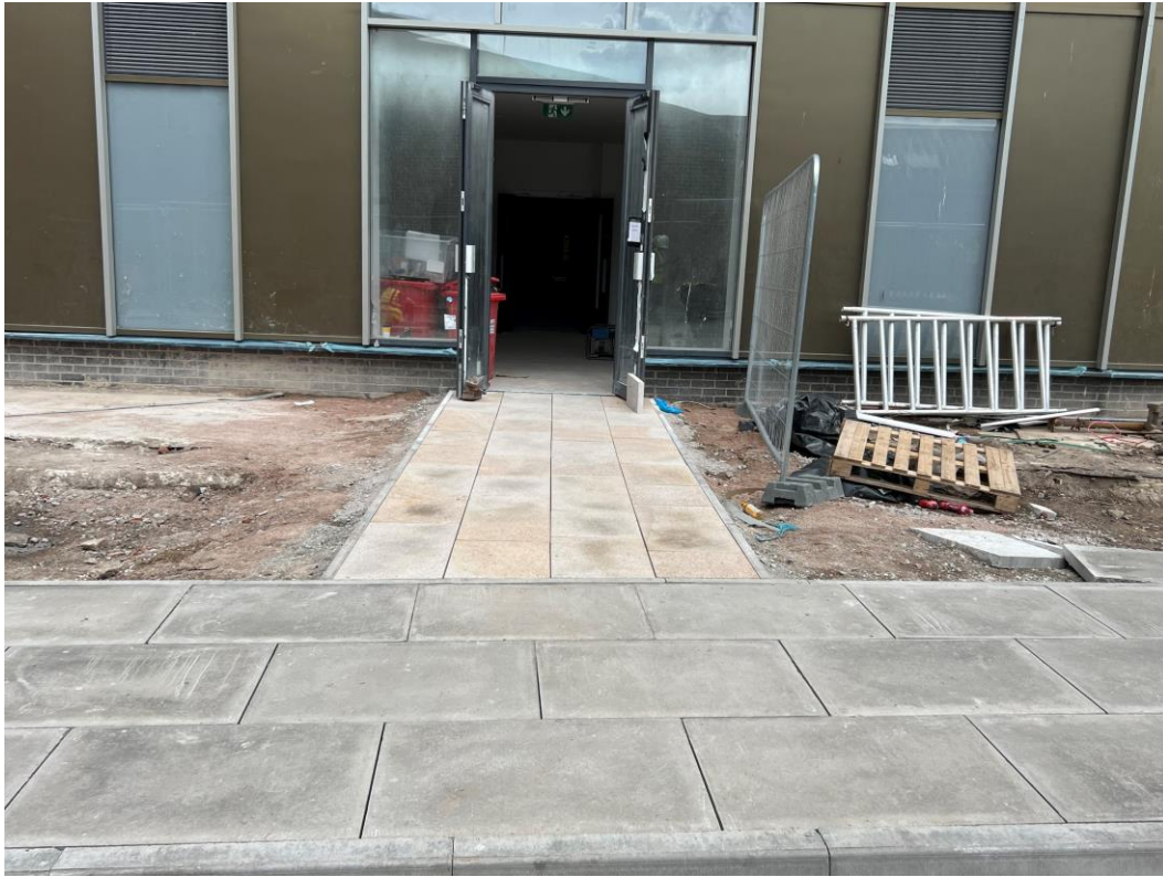
Paving ongoing to Brindley Street elevation
