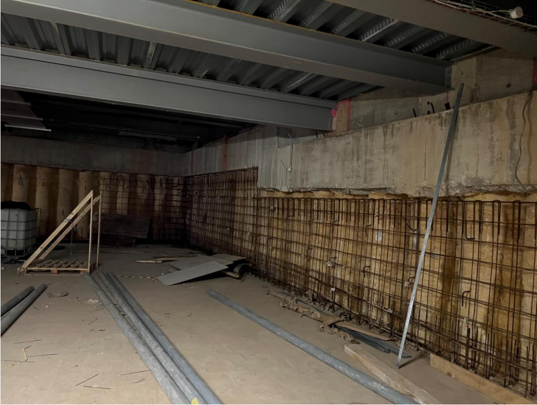
Concrete infill ongoing to basement area
