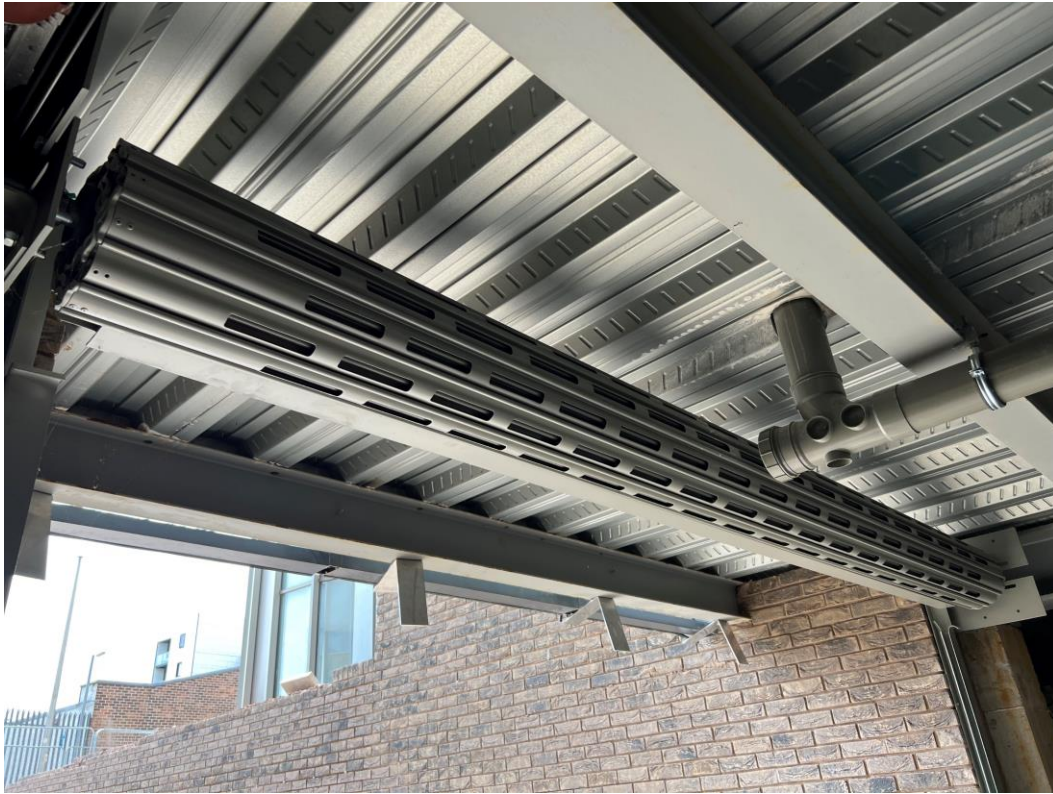
Roller shutters installed to basement ramp
