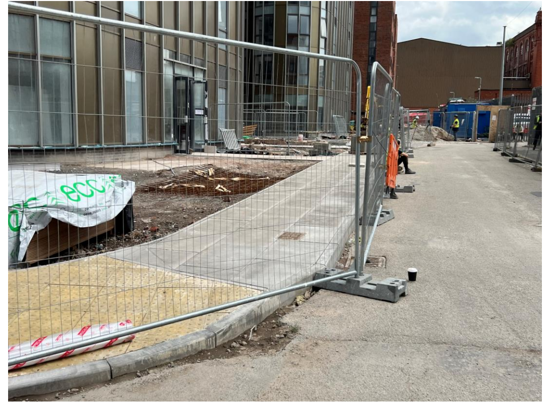
Paving ongoing to Brindley Street elevations
