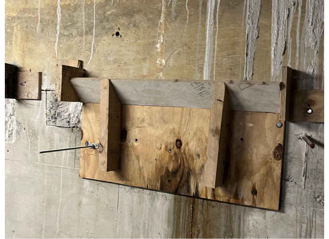
Shuttering installed for concrete infill
