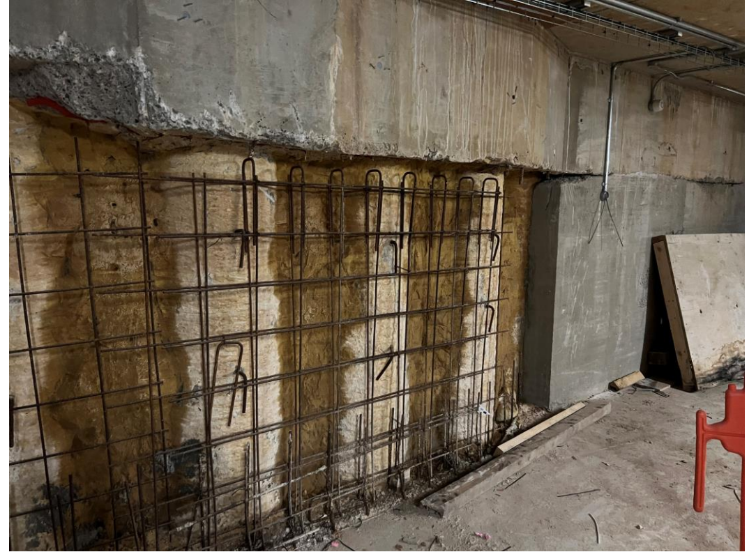
Concrete infill ongoing to basement area
