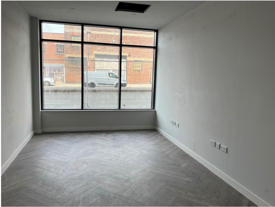
Ground Floor – Finishes to office areas
