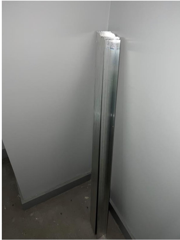
Stair tread nosing's onsite for installation
