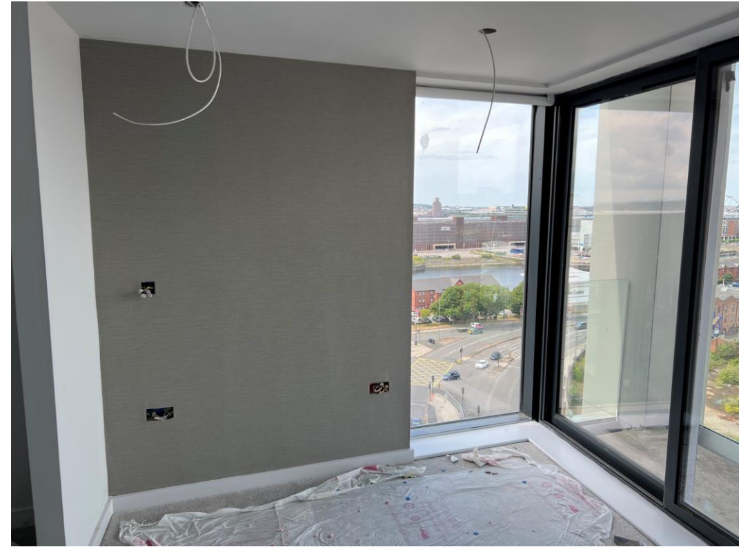
Feature wall installed to bedrooms
