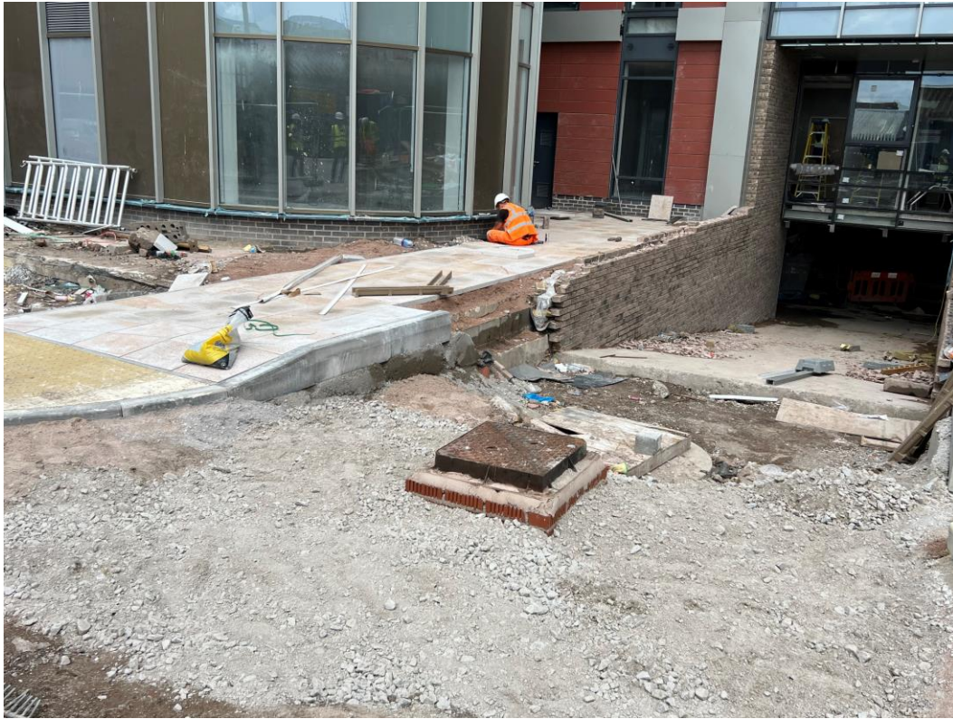
Drainage complete with manhole cover installed
