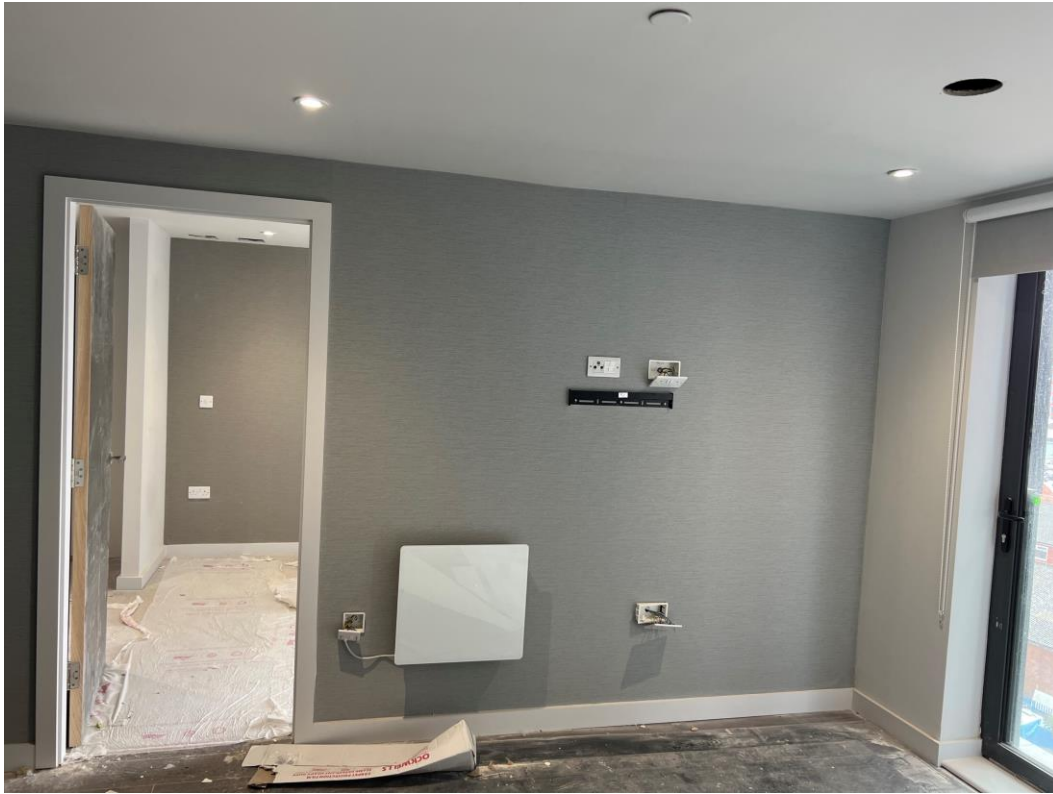
Feature wall installation to lounge
