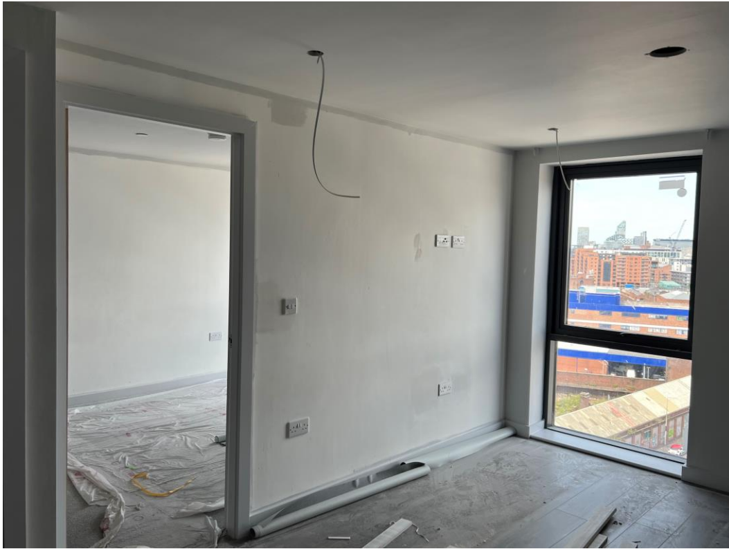
Lounge finishes ongoing
