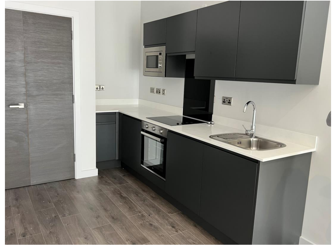
Ground Floor – Kitchen Installed
