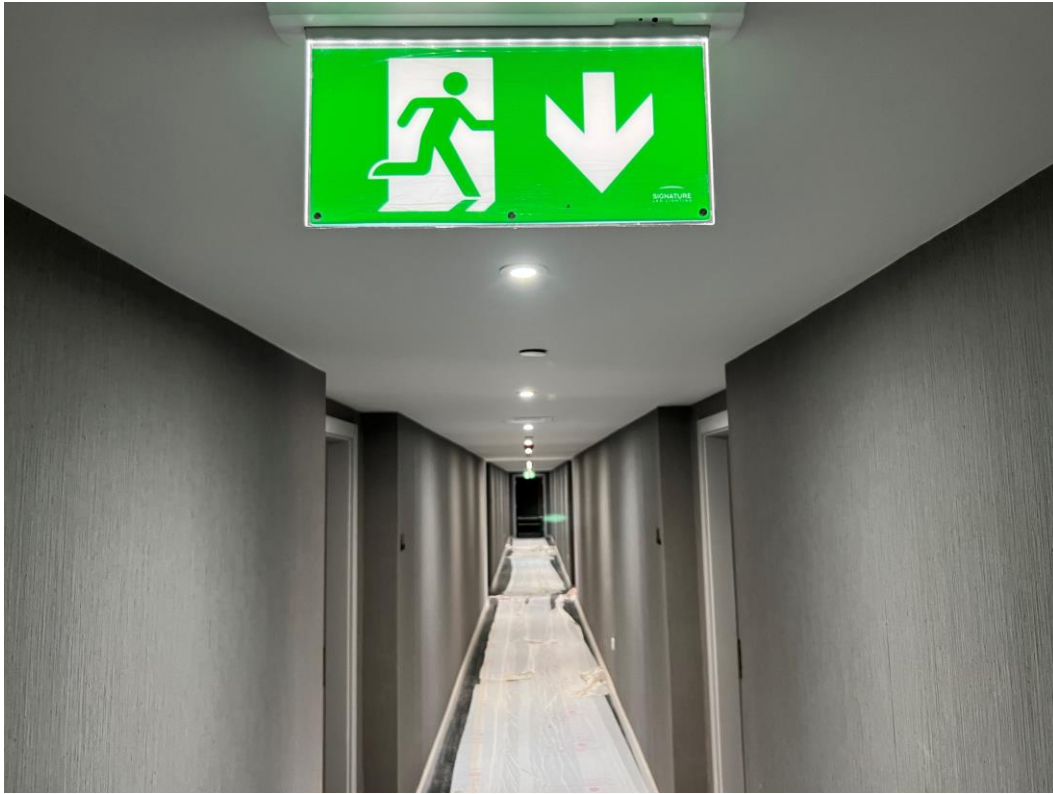
Fire escape signage installed
