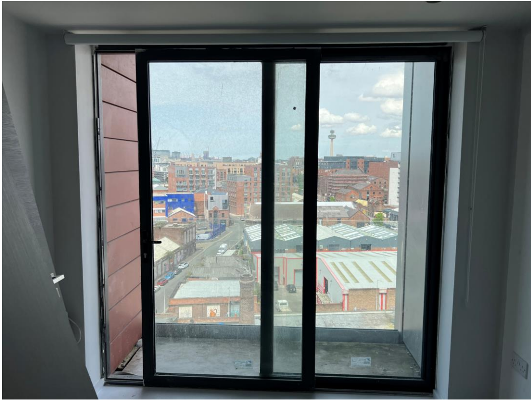
Apartment sliding doors installed
