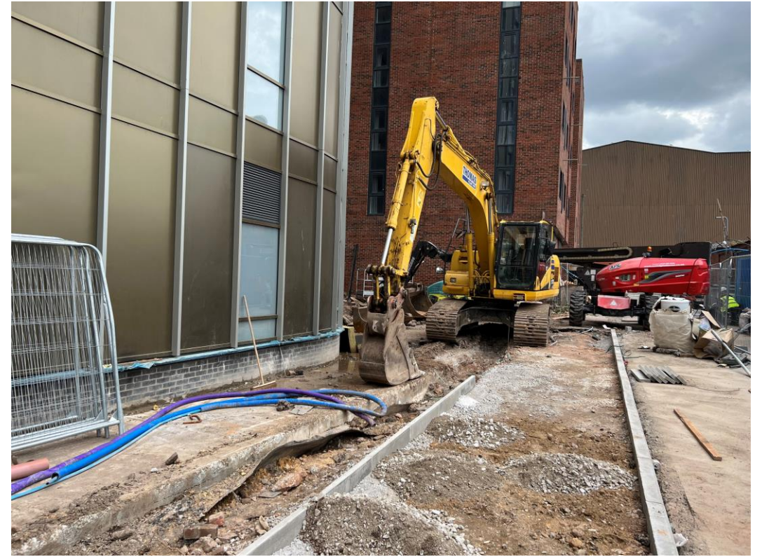
Paving ongoing to Brindle Street elevation
