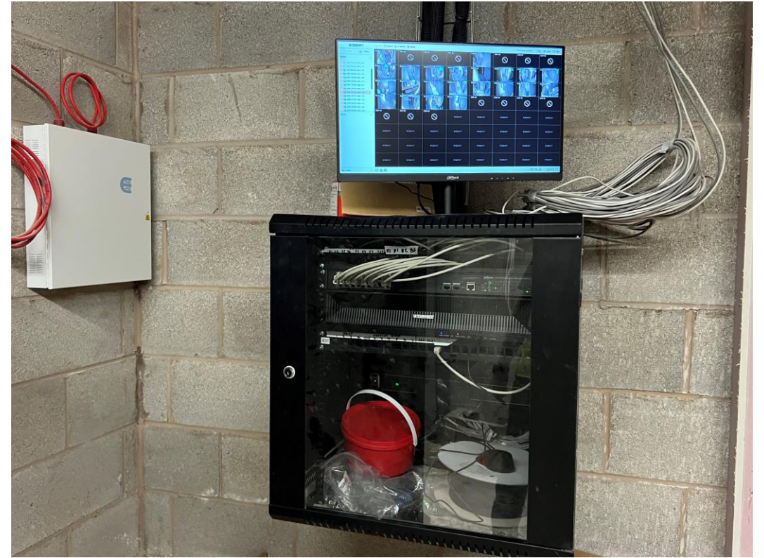
CCTV installation ongoing
