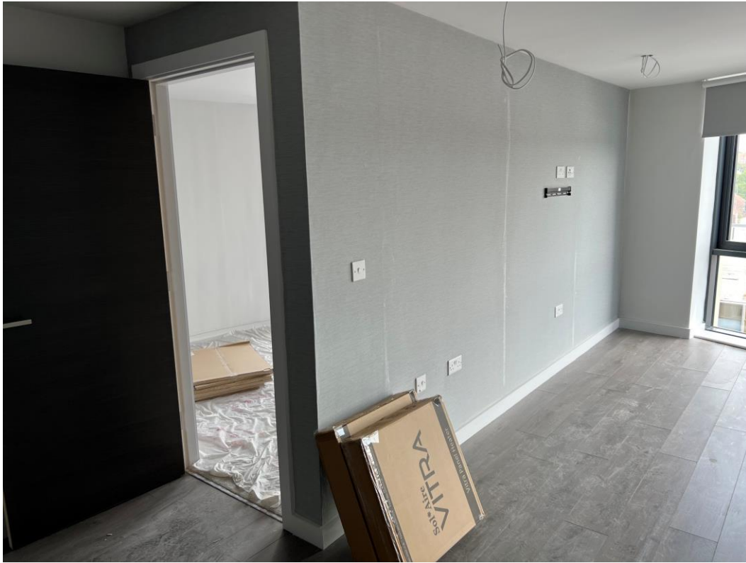
Feature wall installation to lounge
