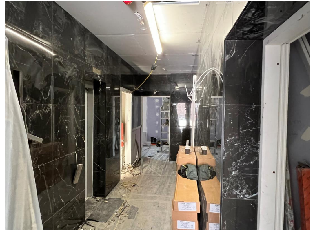
Ground Floor - Finishes to ground floor lift lobby
