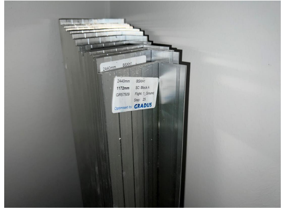
Stair tread nosing's onsite for installation
