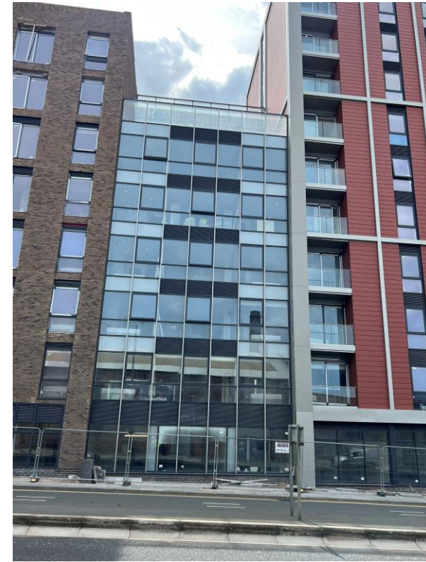
Glazed Balustrades installed to apartment balconies
