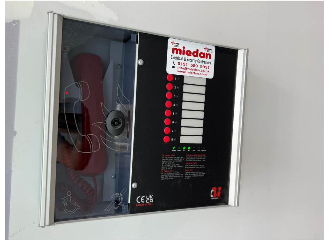
Ground floor - Lexicomm unit installed
