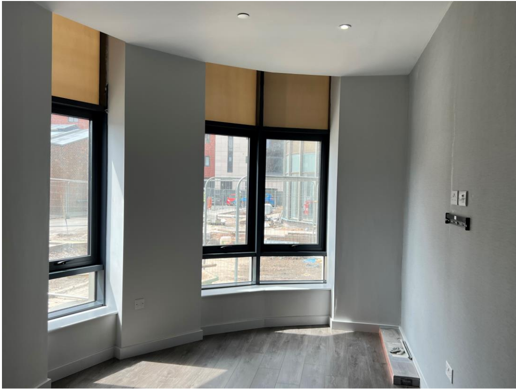
Ground Floor - Apartment lounge finishes
