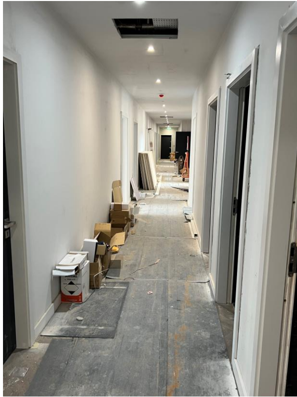
Ground Floor- Circulation area finishes ongoing
