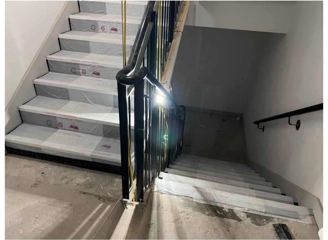
Ongoing finishes to stairwell
