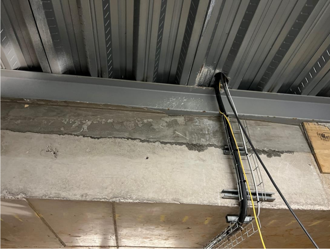
Concrete infill ongoing to basement area
