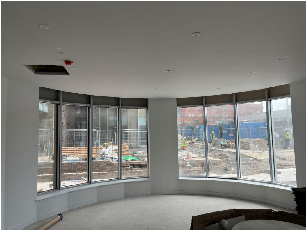
Ground Floor - Finishes to gym area ongoing
