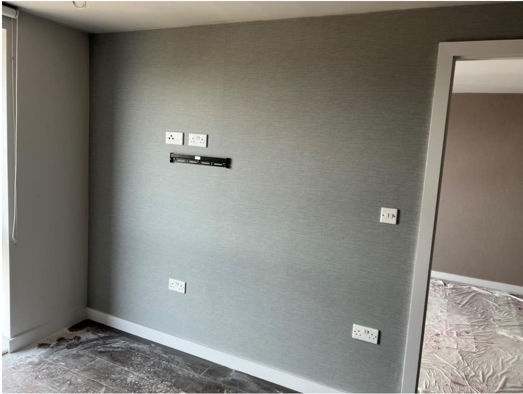
Feature wall installation to lounge
