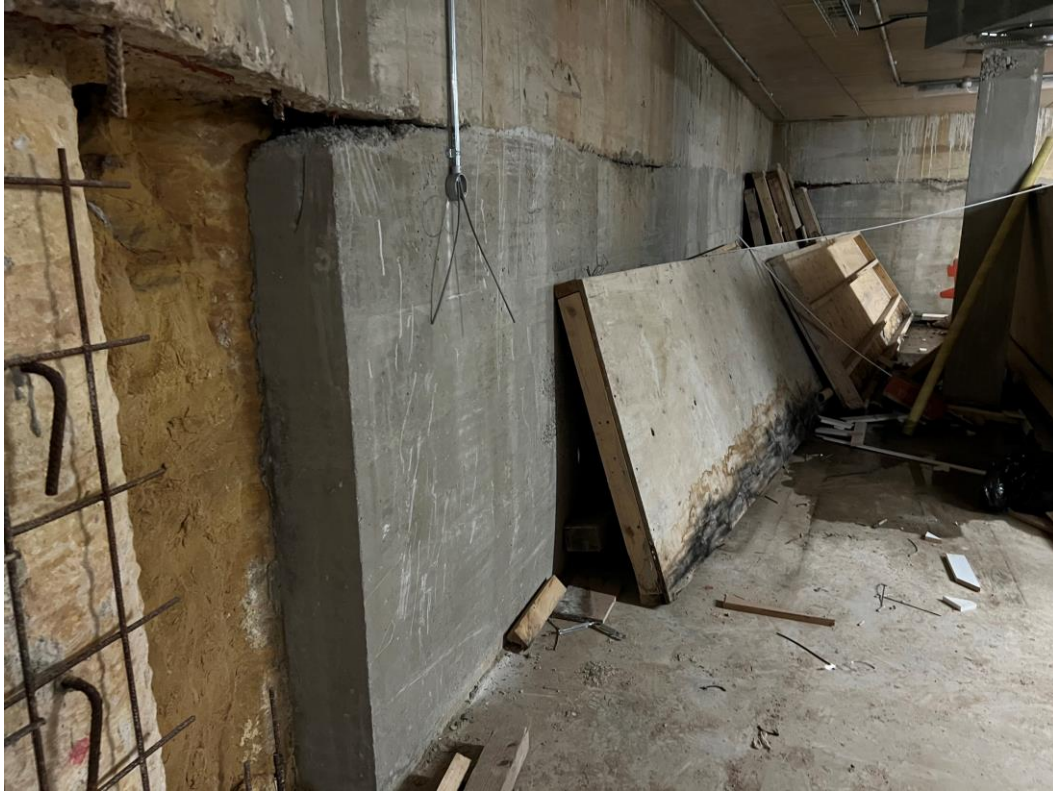
Concrete infill ongoing to basement area
