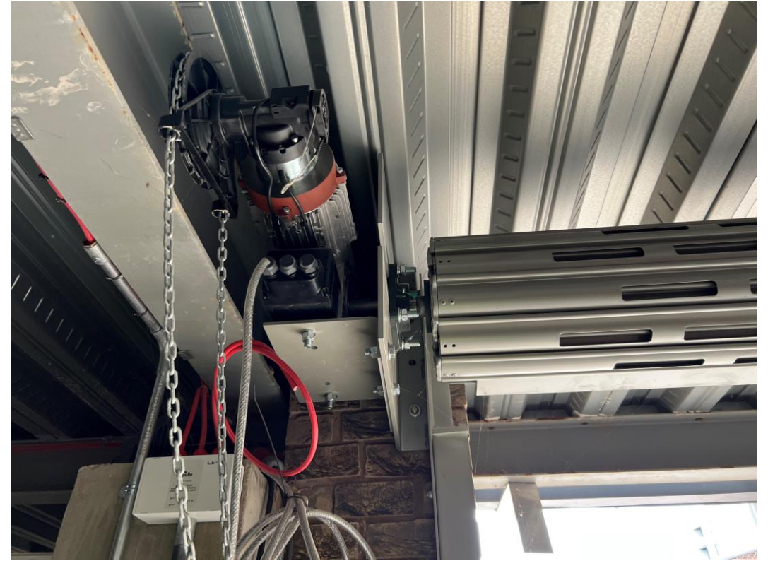
Roller shutters installed to basement ramp
