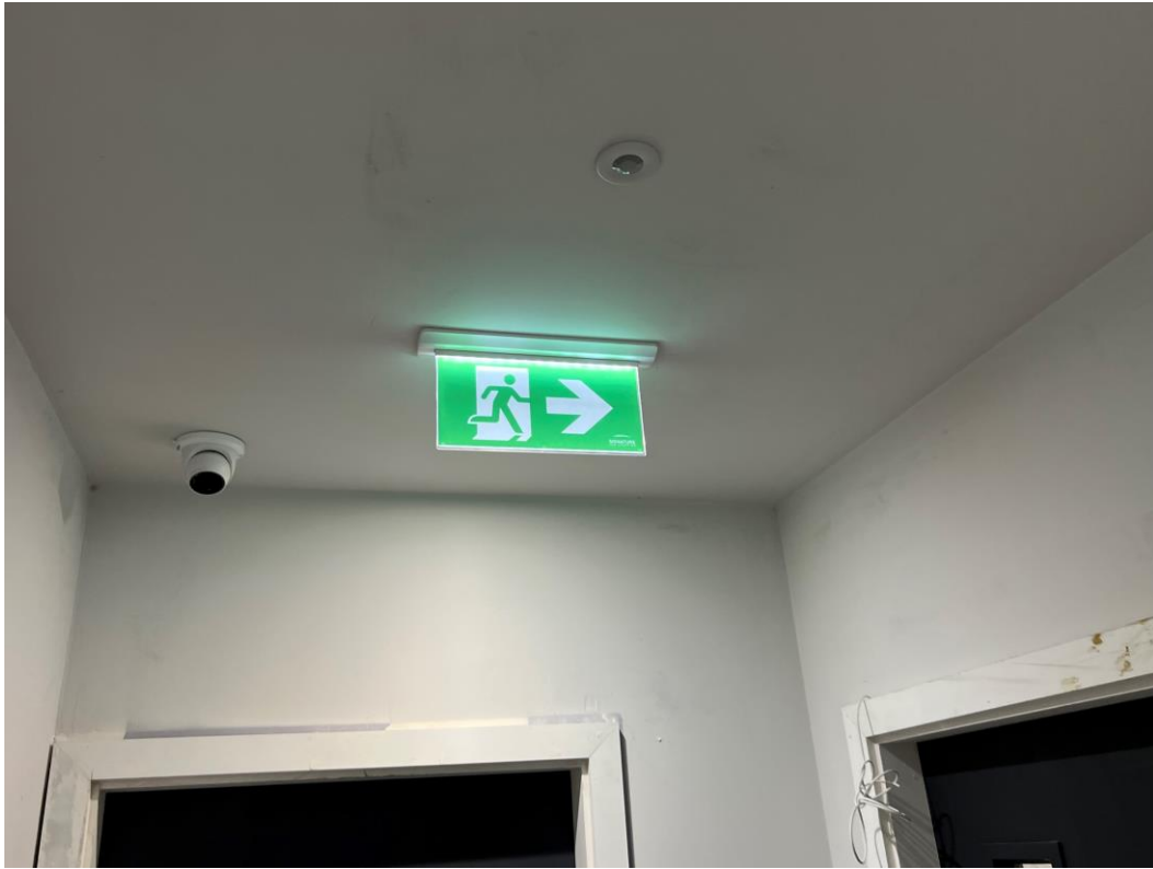
Fire exit signage installed
