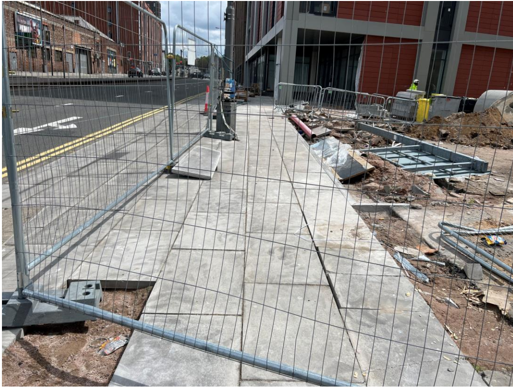
Paving to Parliament Street ongoing
