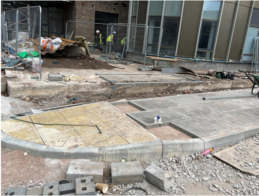
Paving ongoing to Brindle Street elevation
