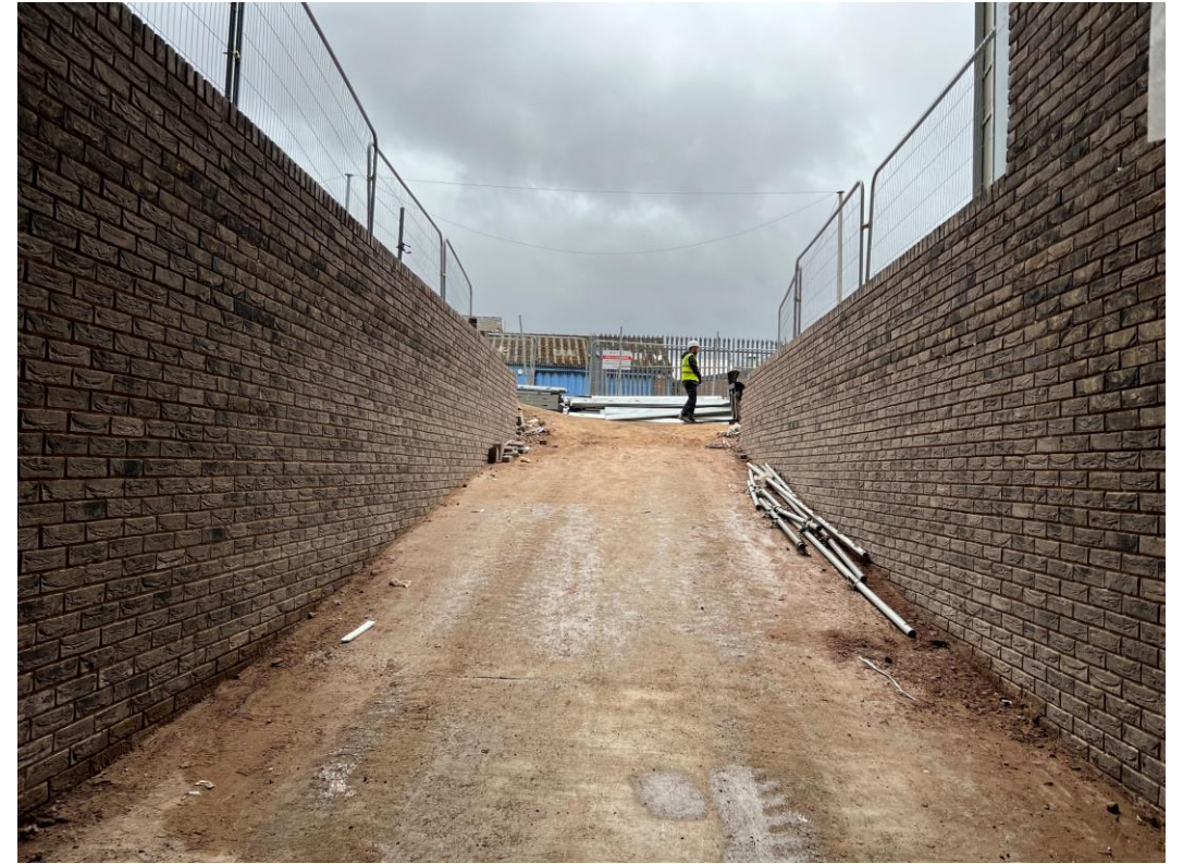
Brickwork installation to basement ramp
