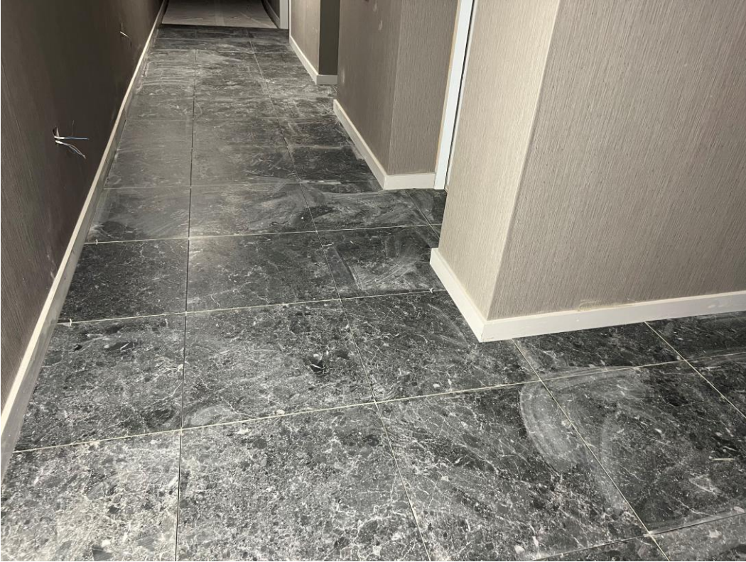
Lift lobby floor tiling
