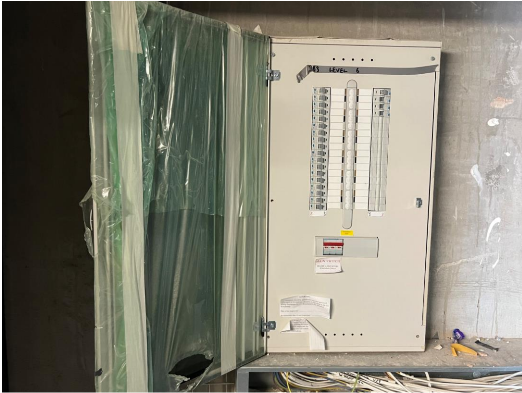
Electrics consumer unit installed
