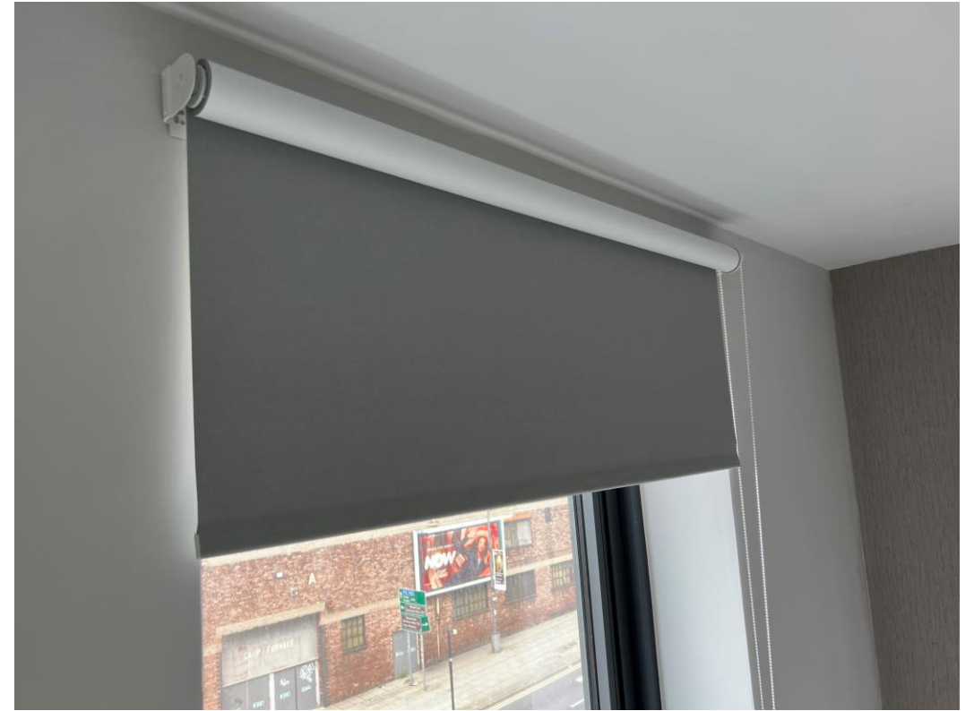
Apartment blinds installed
