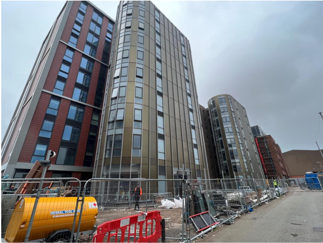
Brindley Street site view
