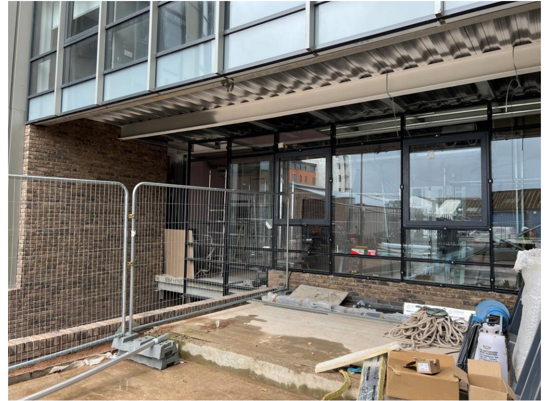
Brindley Street – Window installation
