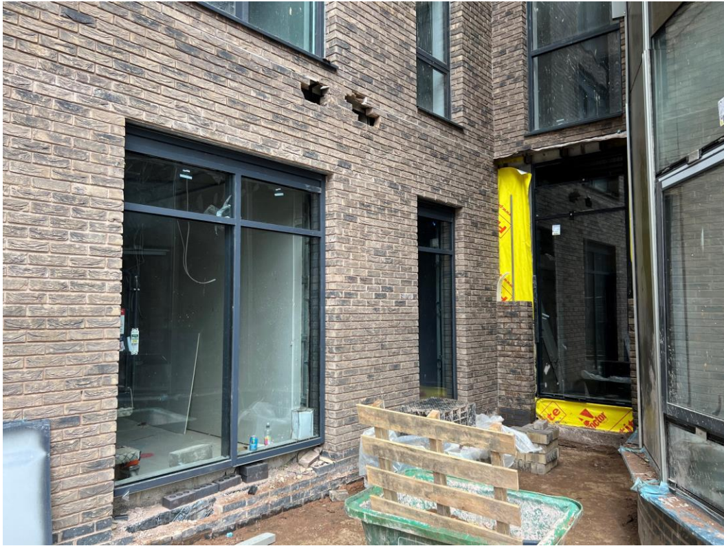
Brindle Street – External brickwork
