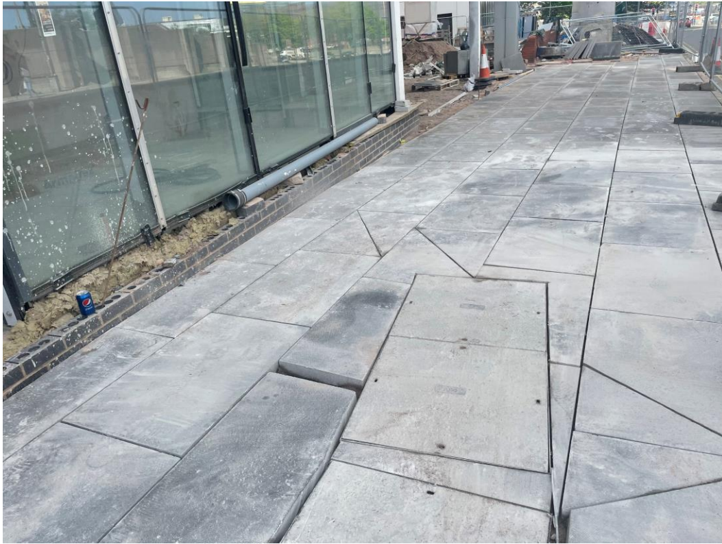
Parliament street –Magma paving installed
