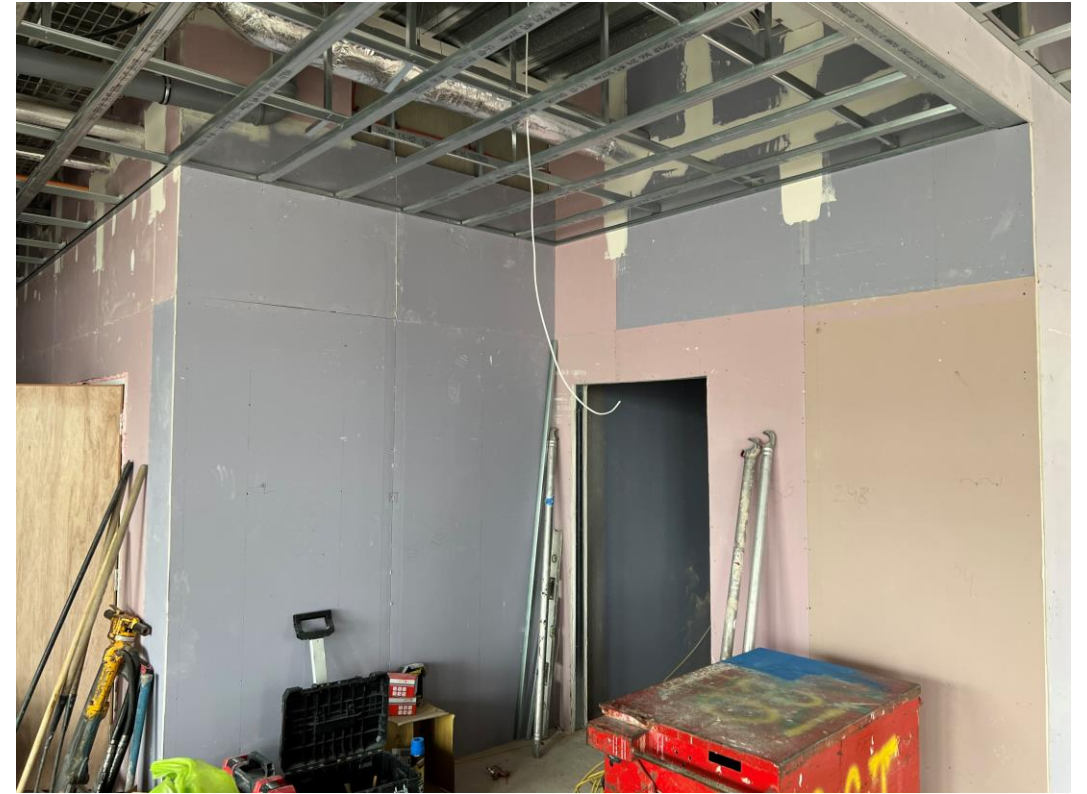
Partitions boarded & ceiling grid erected
