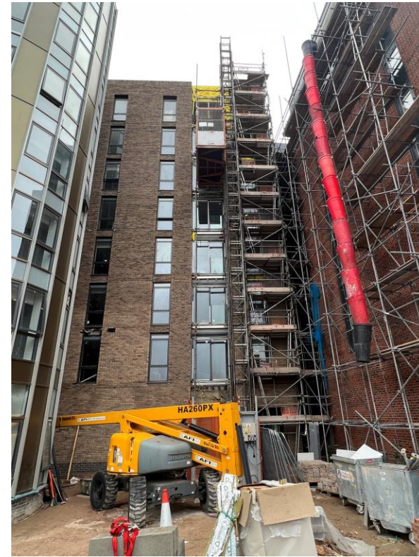
Brindley Street site view
