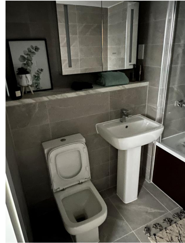
Show Flat – Bathroom Sanitary Items
