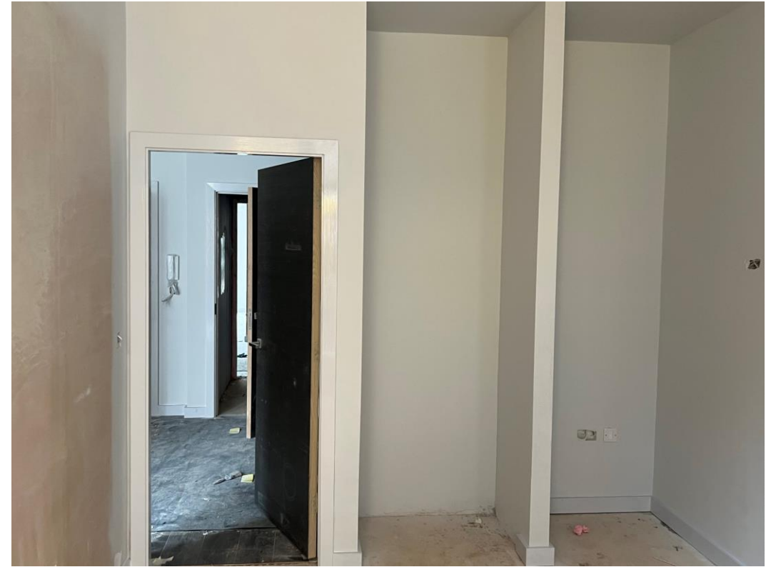
Ground Floor Apartments – internal doors installed
