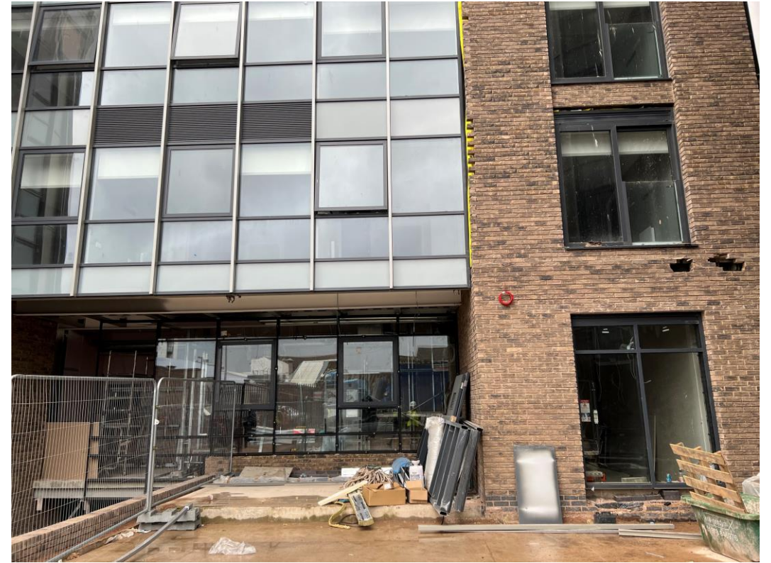
Ground Floor – Window installation ongoing
