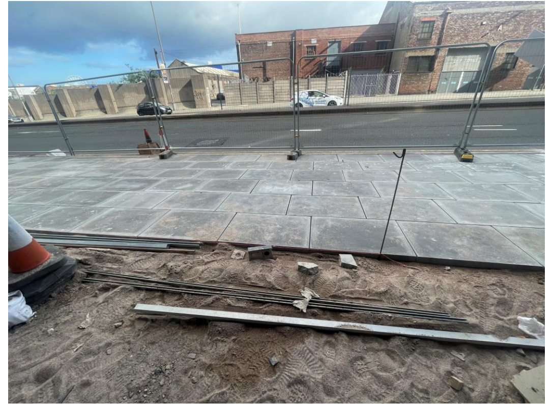
Parliament street –Magma paving installed
