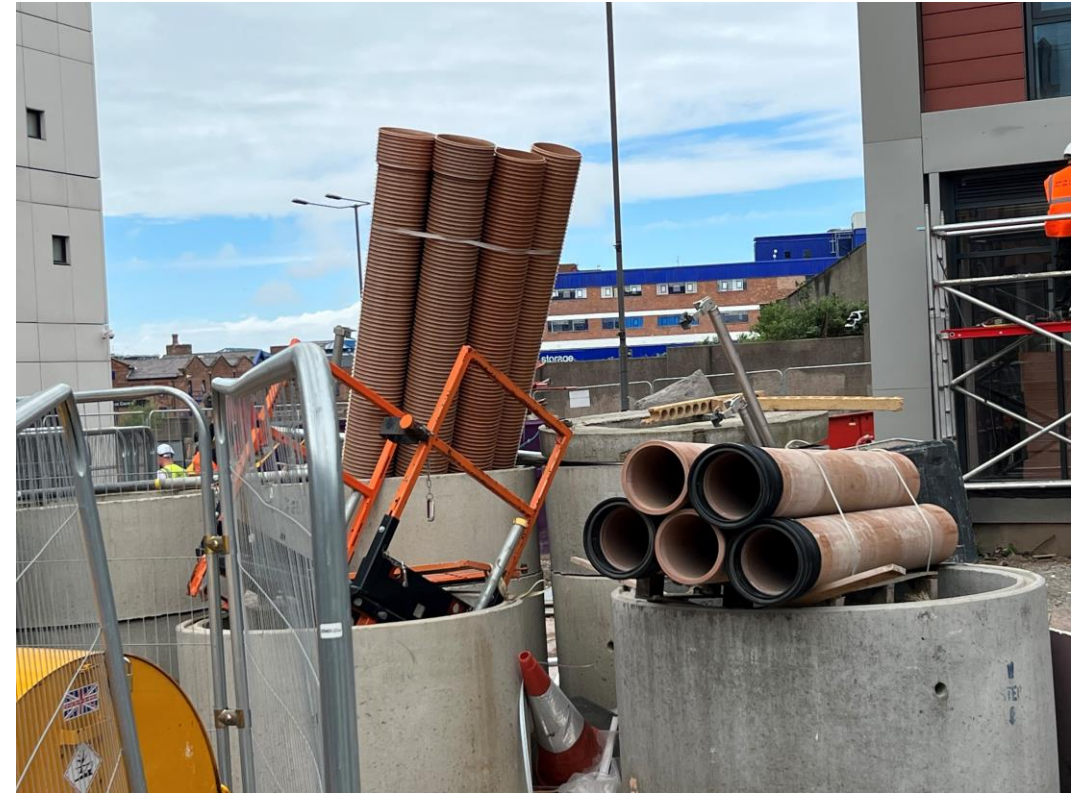
Underground waste pipe onsite for installation
