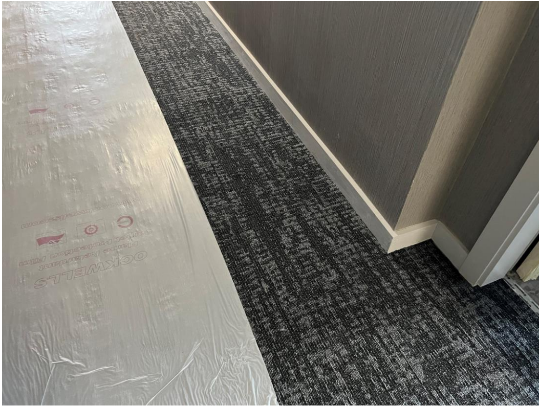
Circulation area carpets installed
