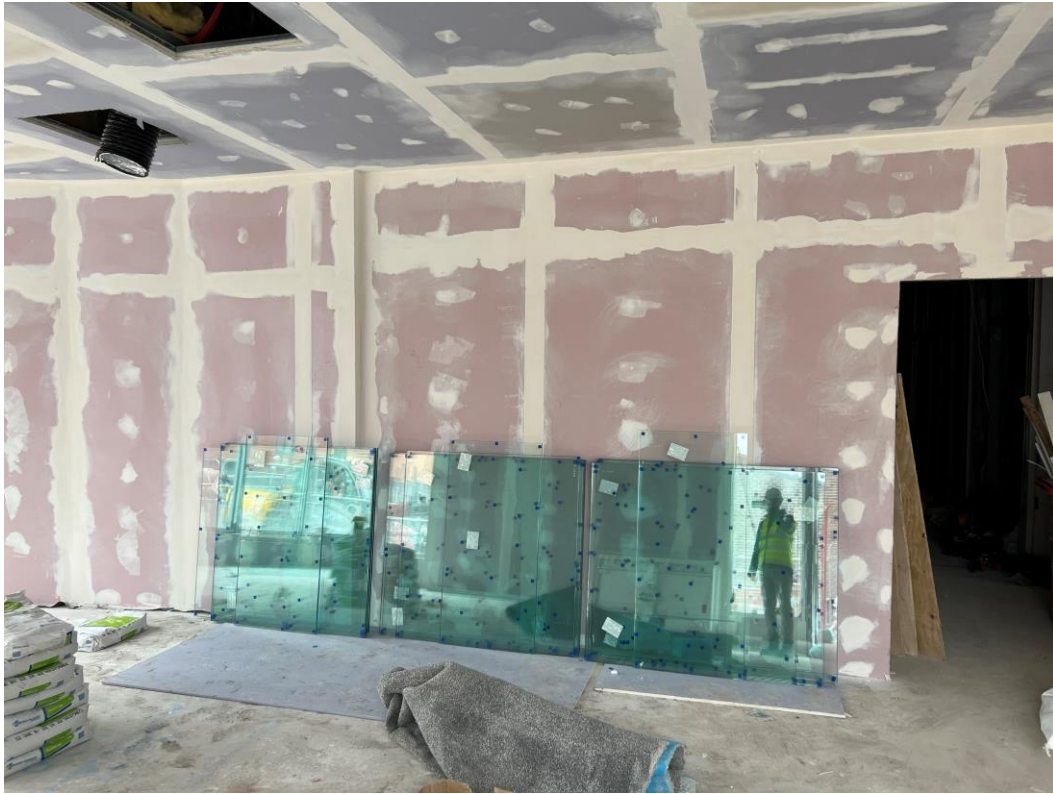
Ground Floor – Gym area tape & jointed
