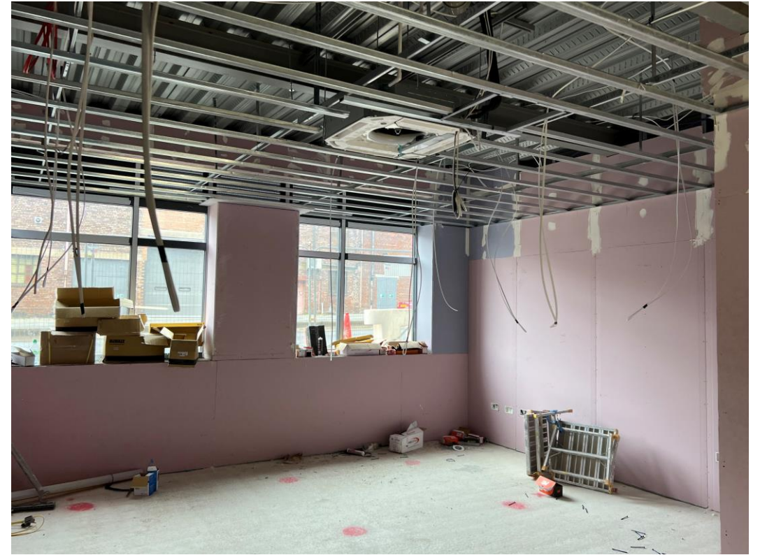
Electrical cable onsite for installation
