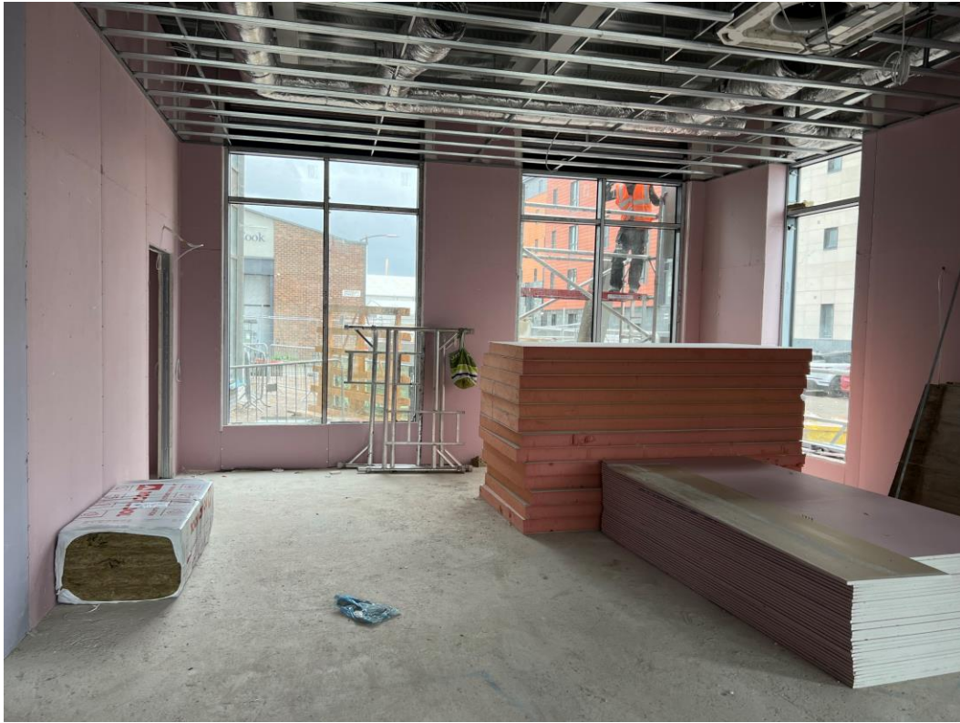
Partitions boarded & ceiling grid erected
