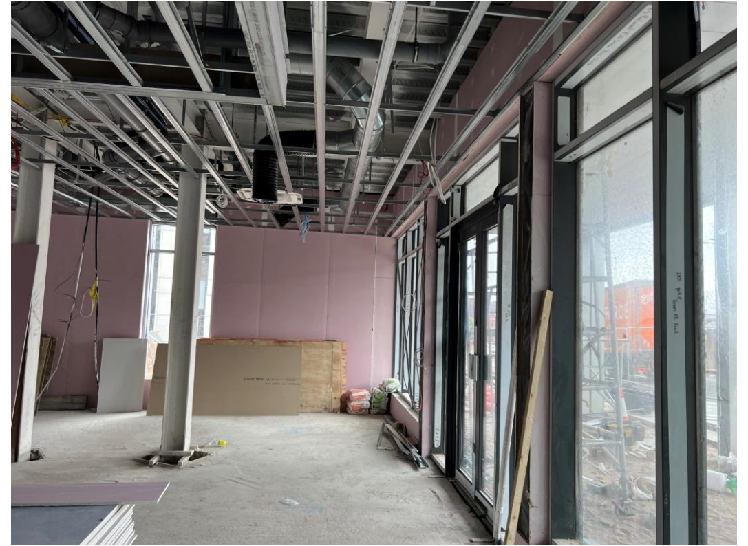
Partitions boarded & ceiling grid erected
