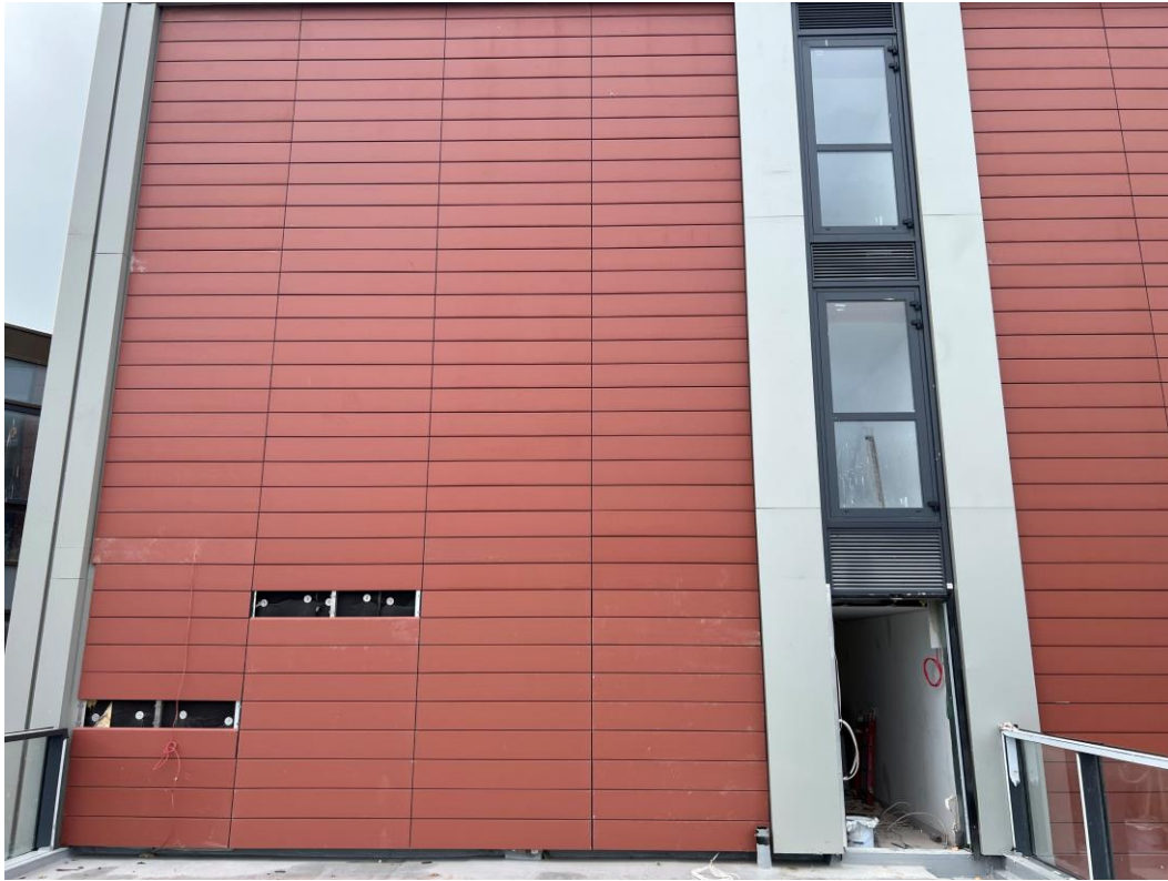
Cladding remedial works
