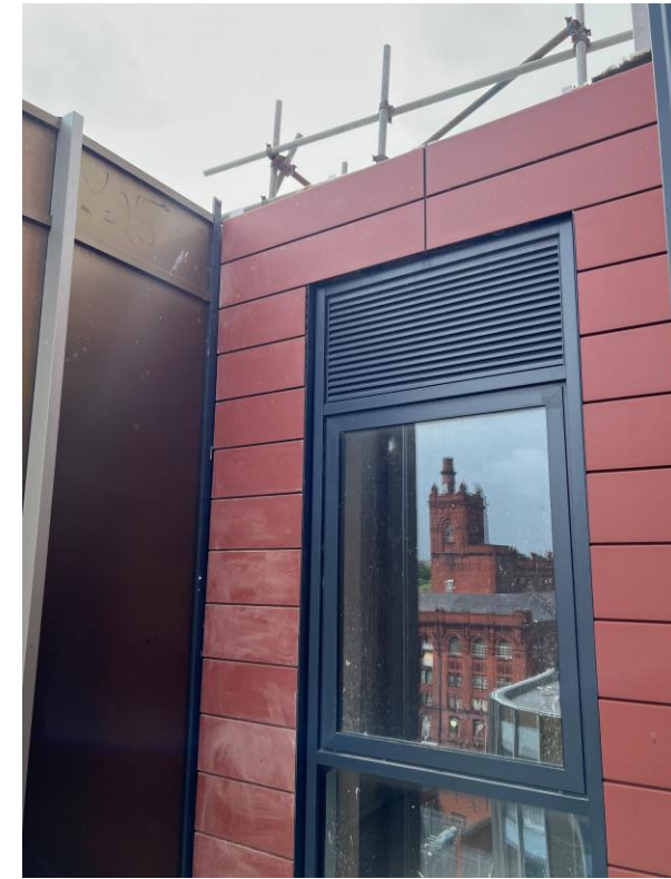
Cladding remedial works
