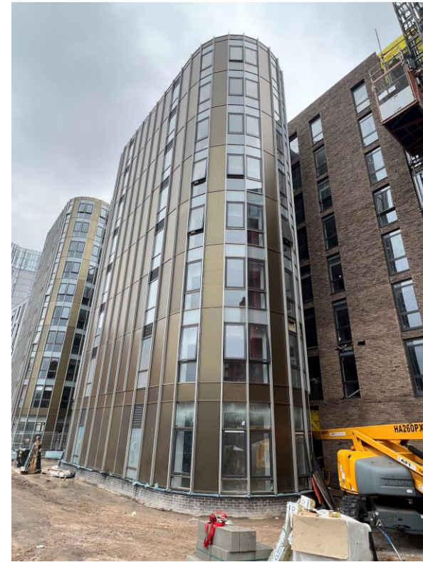
Brindley Street site view
