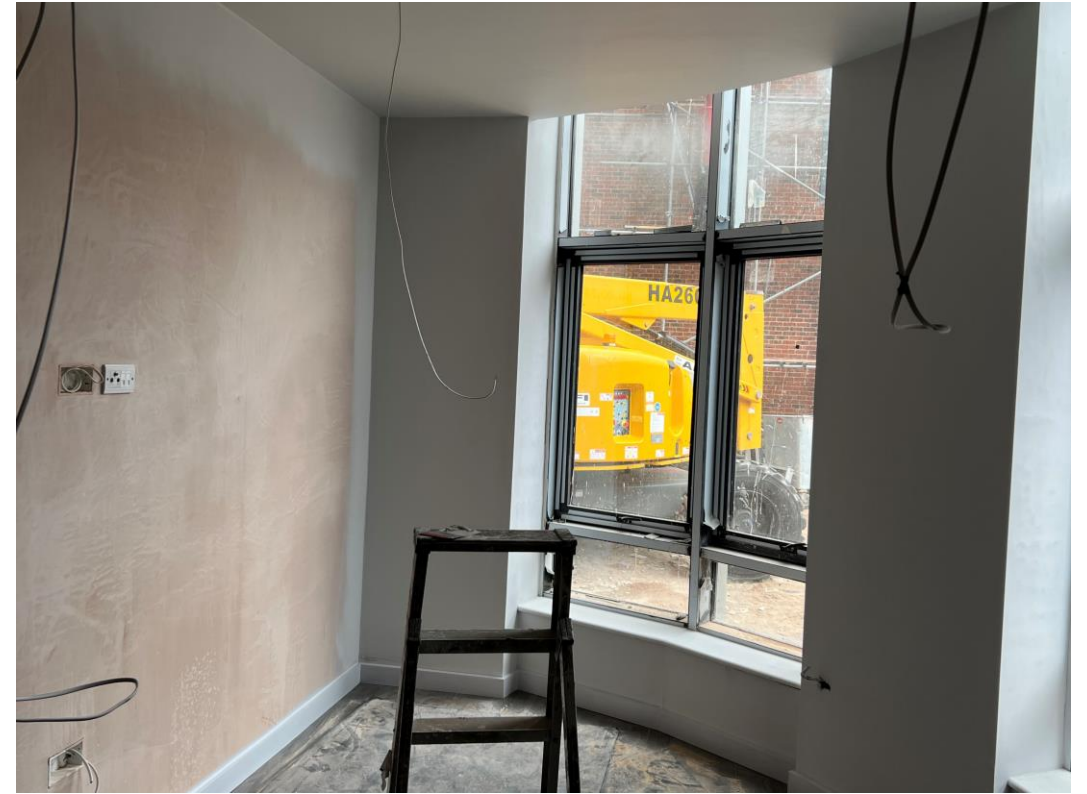
Ground Floor Apartments – Walls & ceilings decorated
