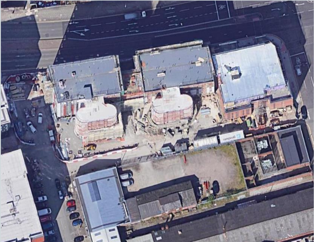
Aerial view of The Summit site location
