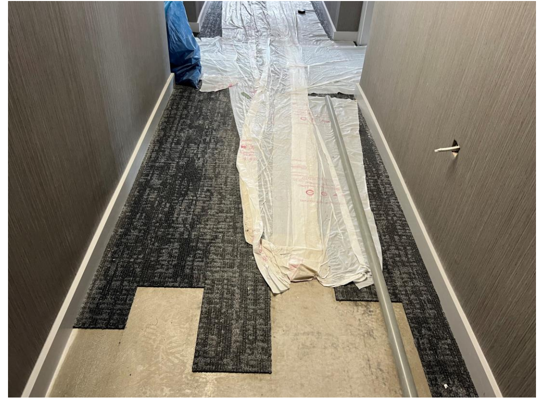
Circulation area carpets installed
