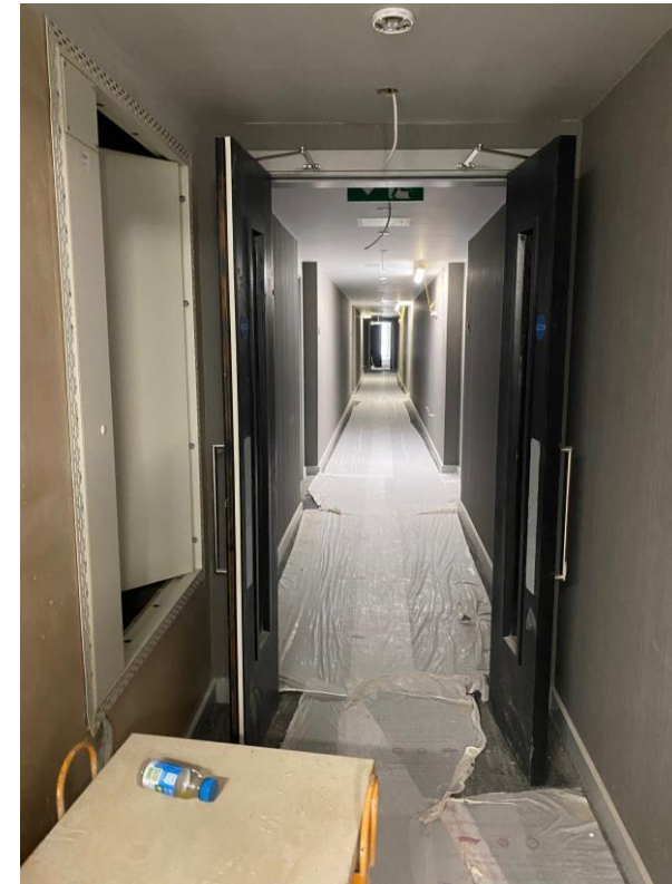
Circulation area fire doors
