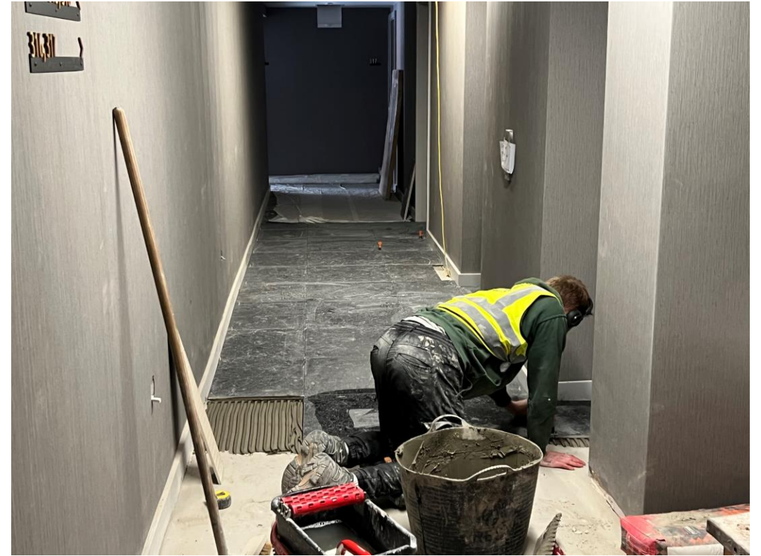
Lift lobby floor tiling
