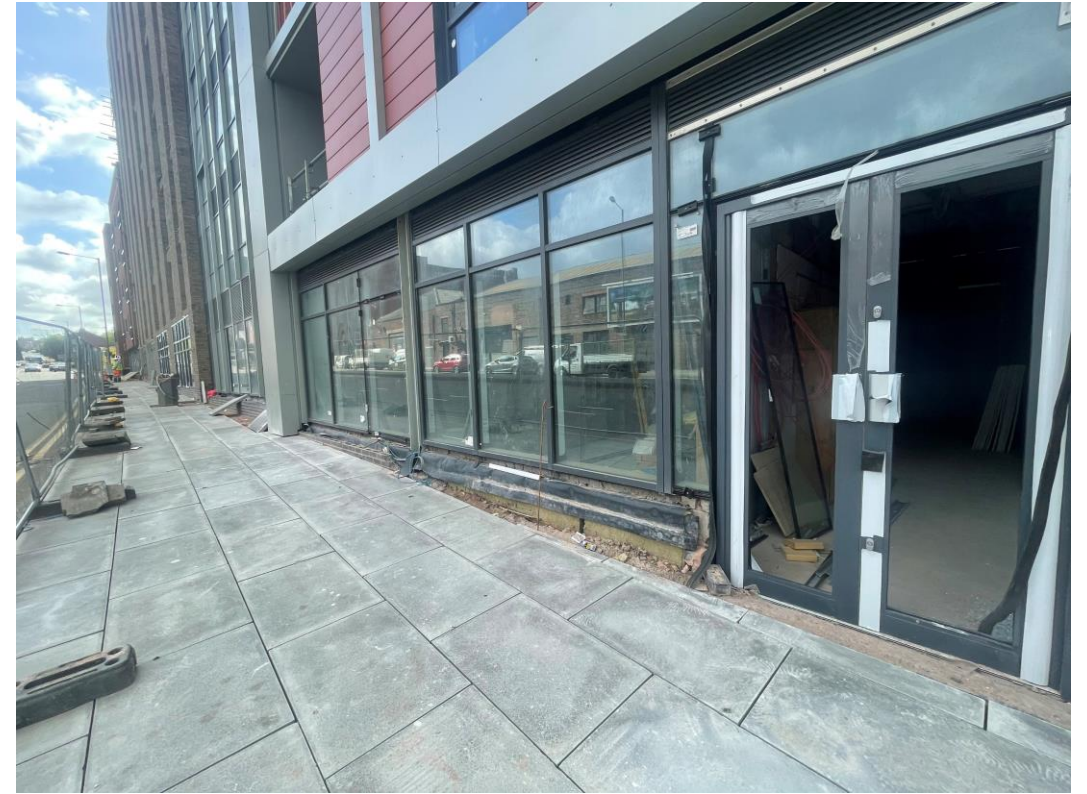
Parliament street –Magma paving installed
