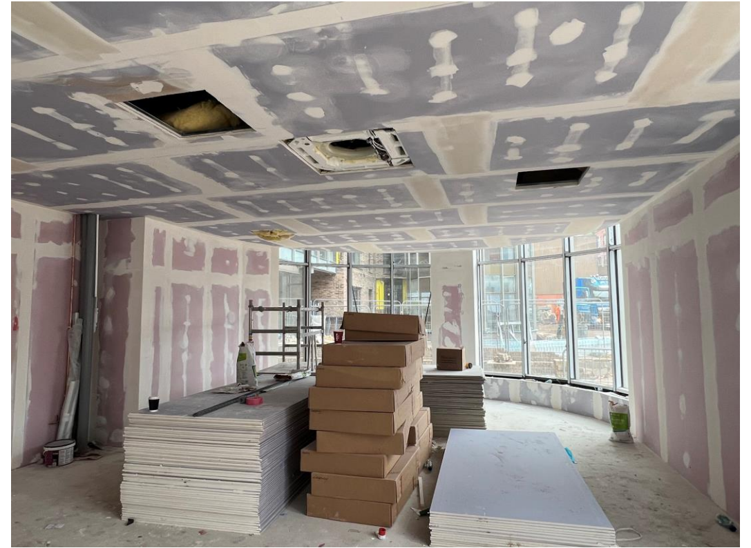
Ground Floor – Gym area tape & jointed
