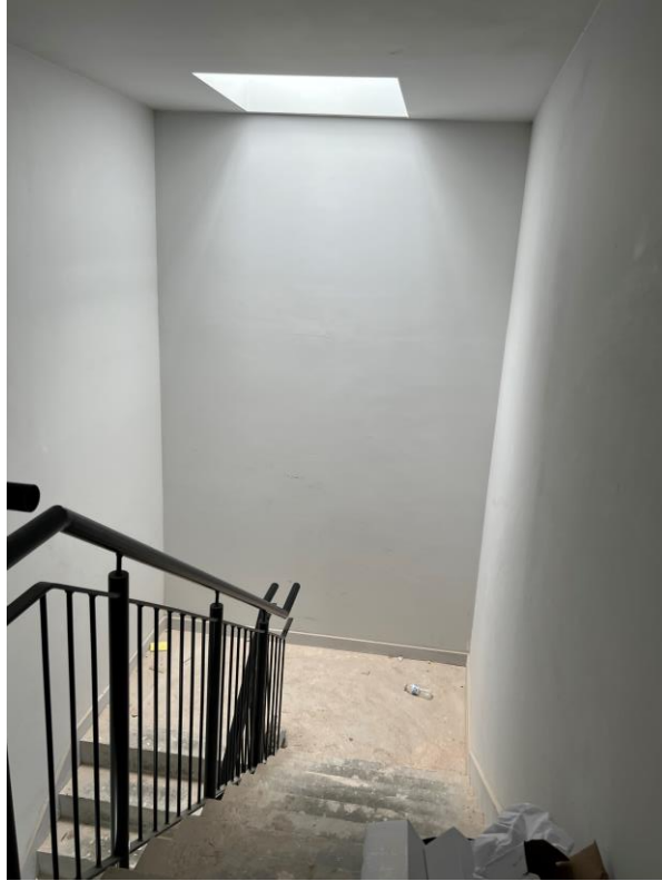
Stairwell decoration ongoing
