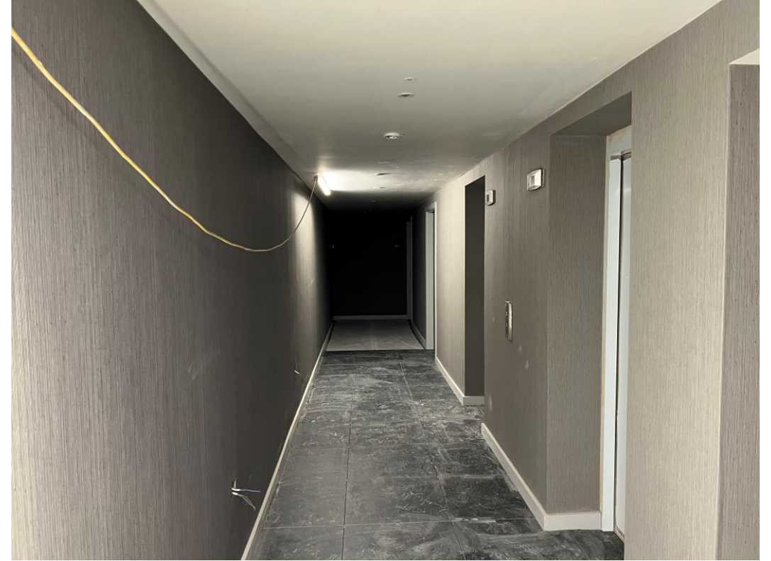
Lift lobby floor tiling
