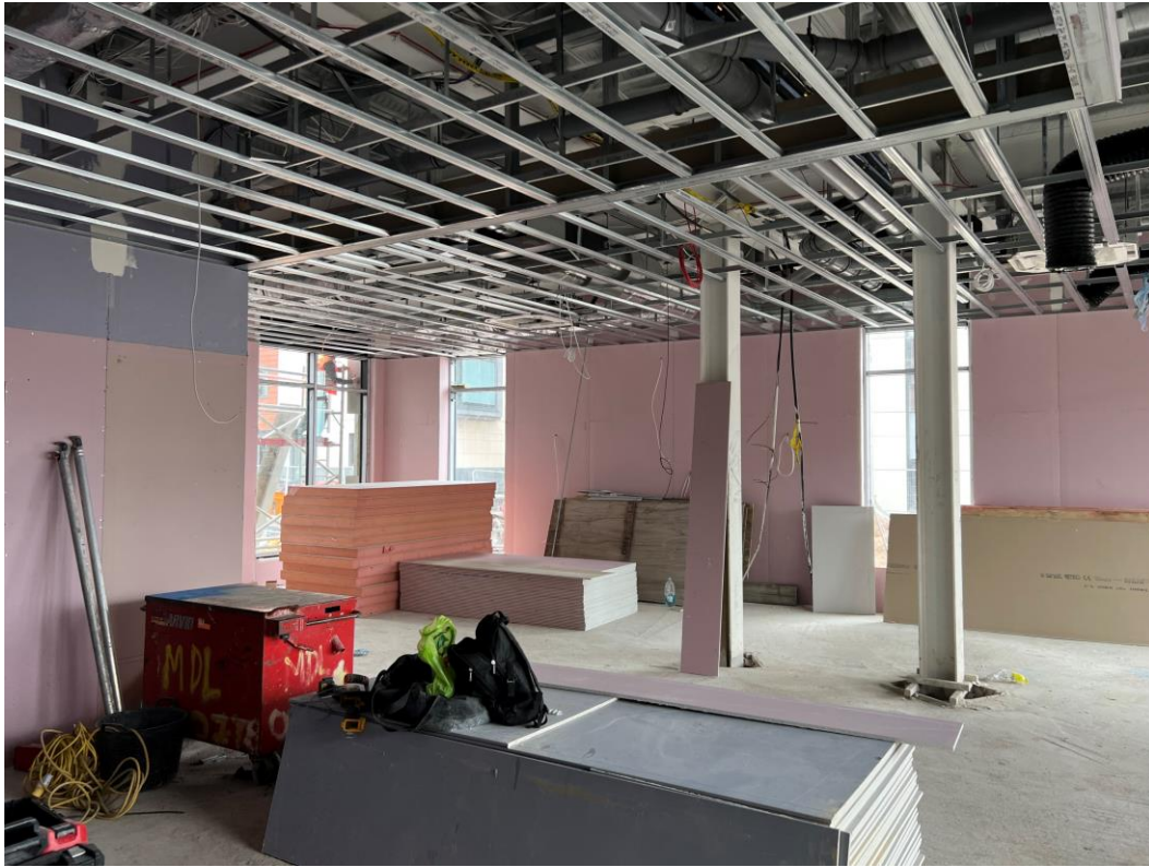
Partitions boarded & ceiling grid erected
