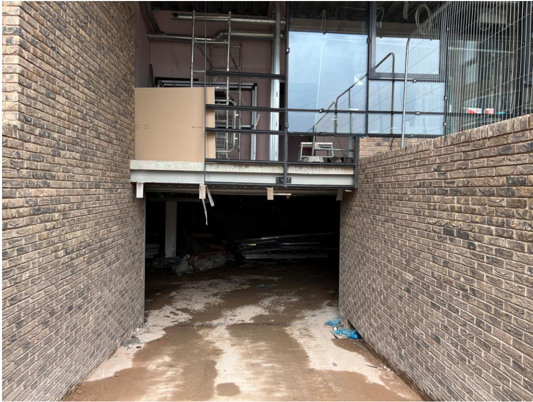
Brickwork installation to basement ramp
