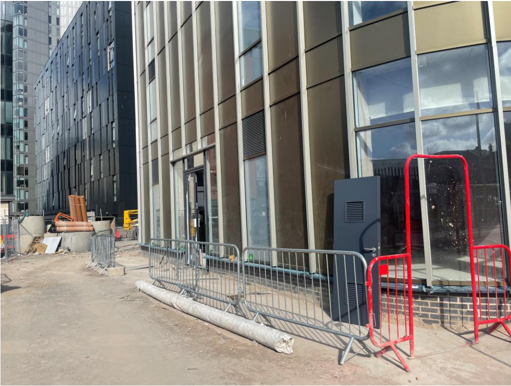
Brindley Street site view
