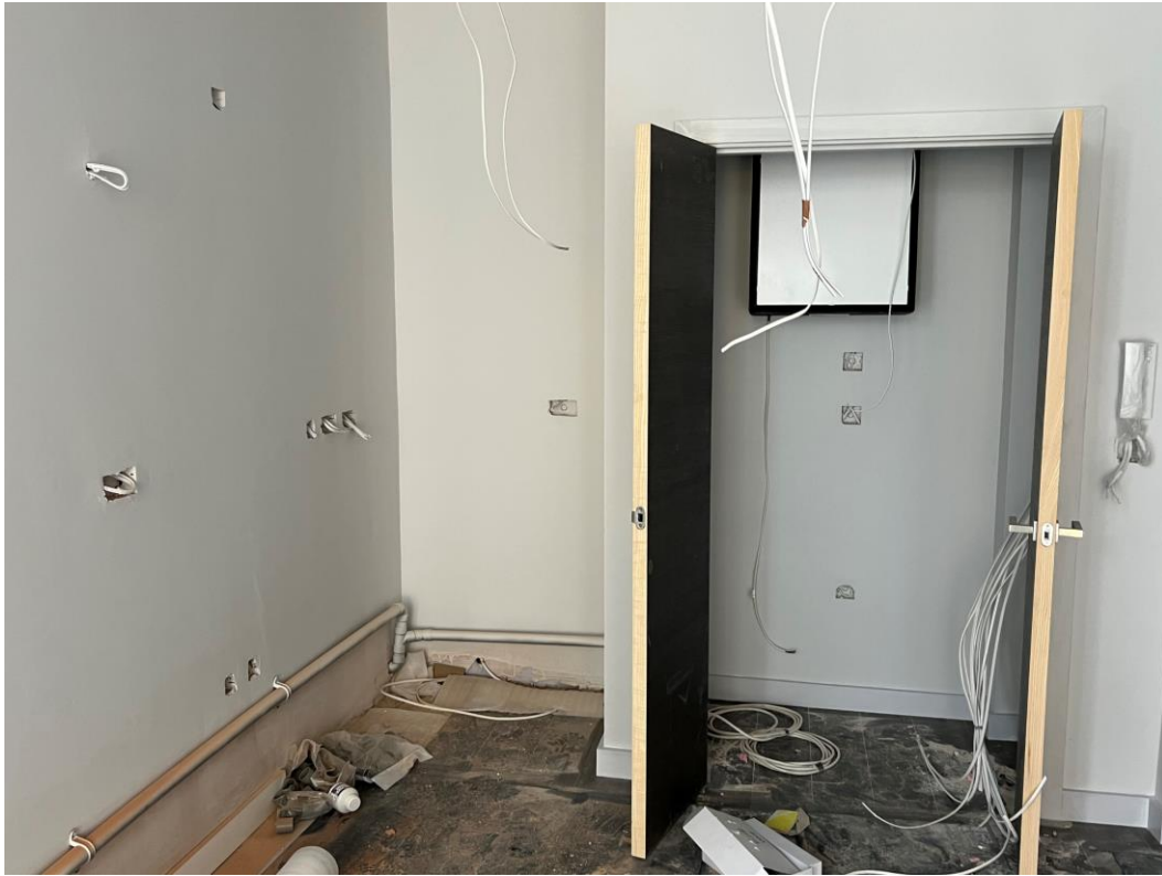
Ground Floor Apartments – 2 nd fix electrics
