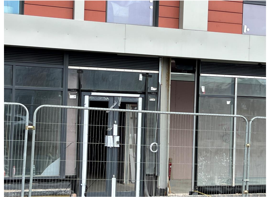
External doors installed
