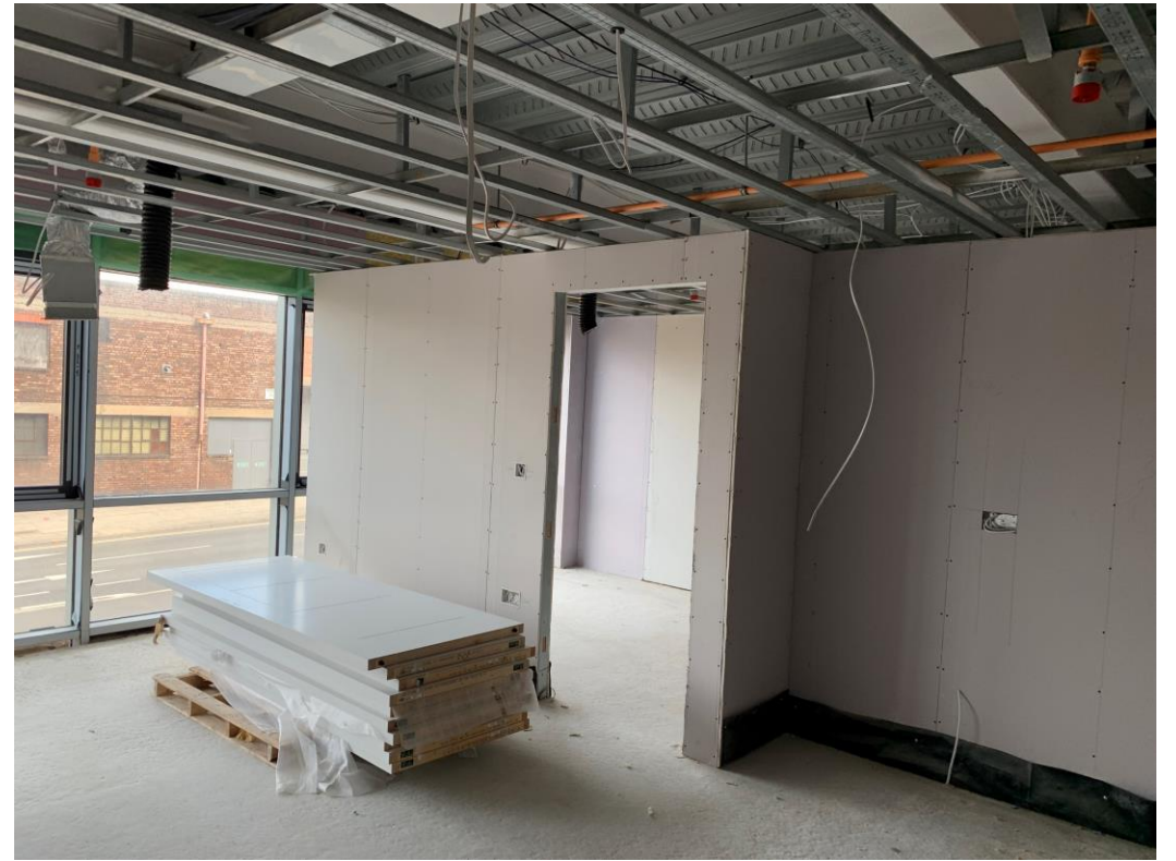
Apartment walls and ceilings under construction
