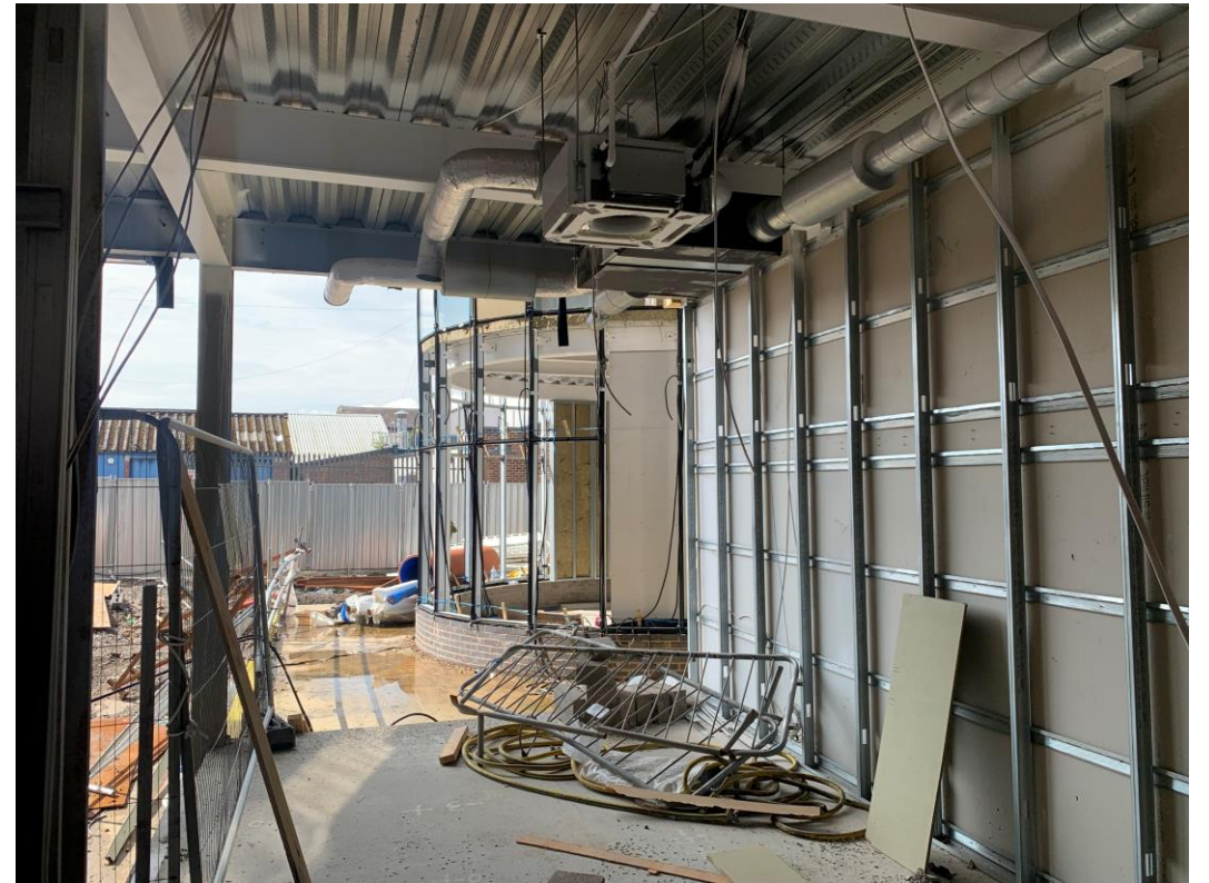
Ground Floor walls and ceilings under construction
