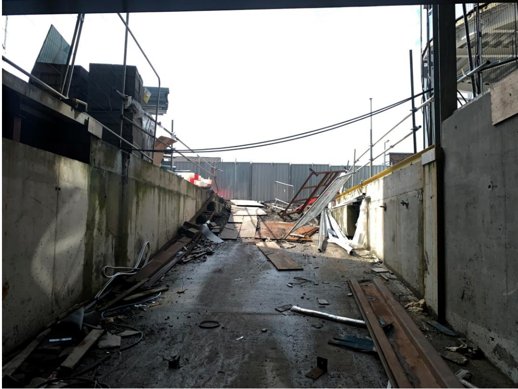
Basement ramp access
