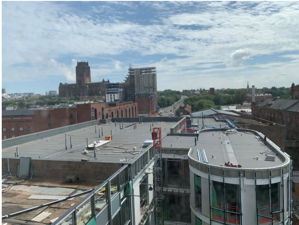
Main flat roof covering
