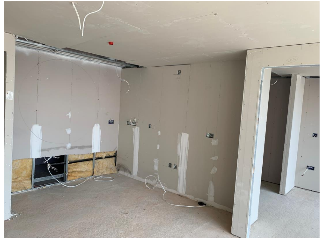
Apartment walls and ceilings boarded
