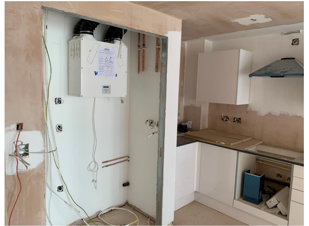
Mechanical ventilation installed / kitchen commenced
