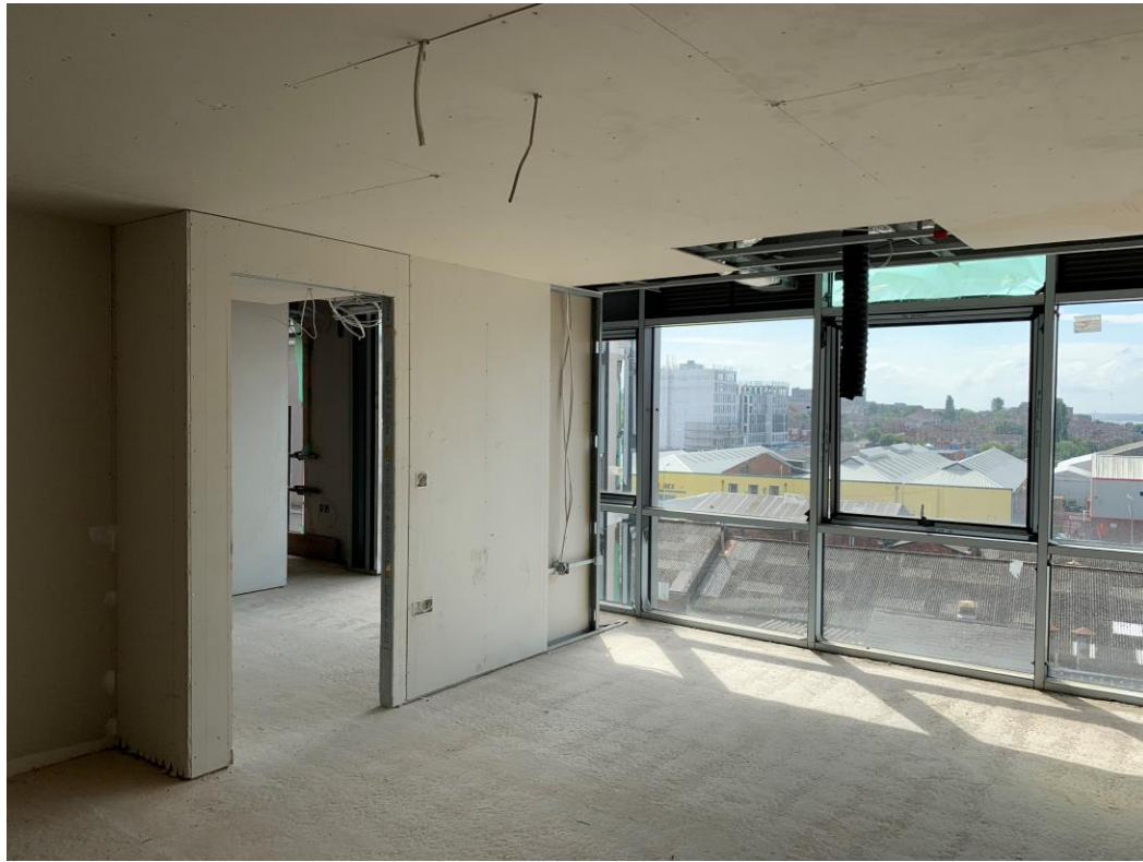
Apartment walls and ceilings boarded
