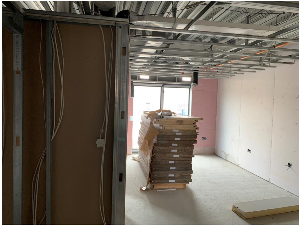
Apartment walls and ceilings under construction
