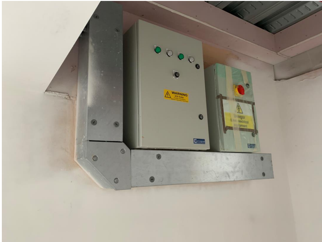
Electrical supply corridor upper floors
