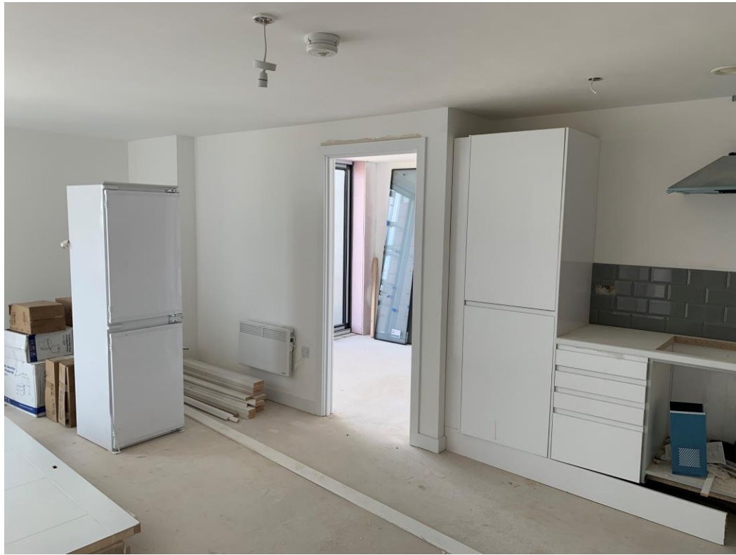
Apartment fitout nearing completion
