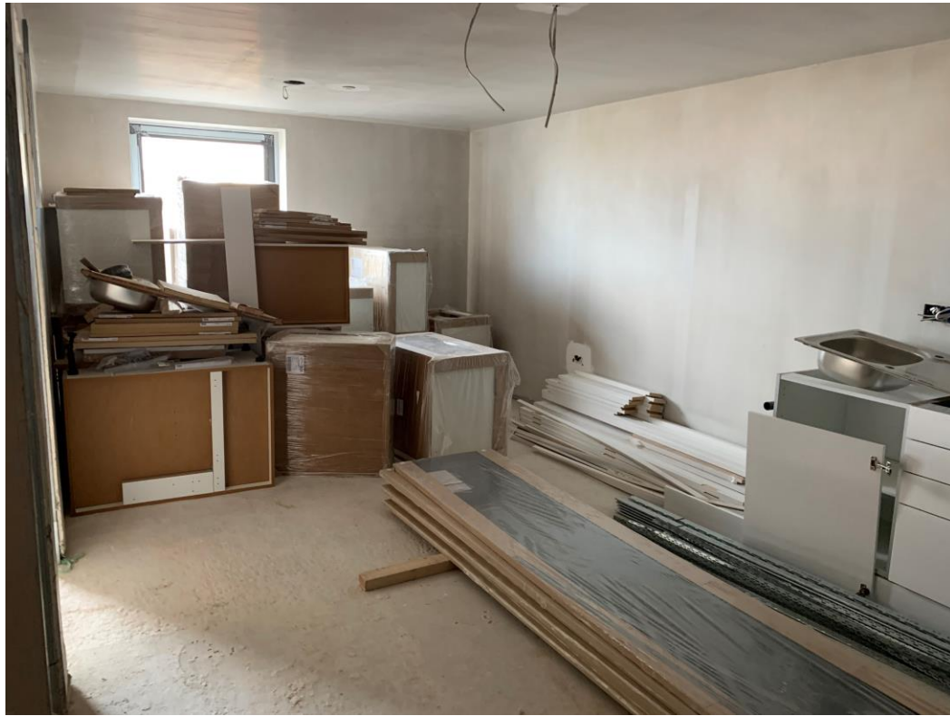
Kitchen loaded for installation
