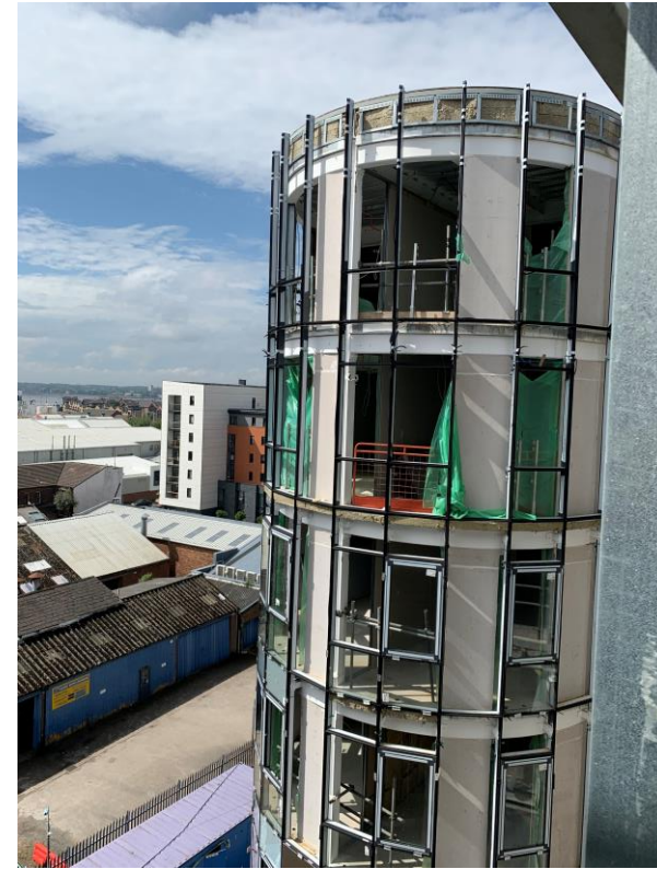
External cladding under construction
