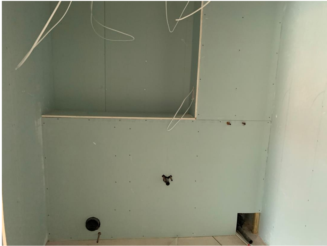
Apartment Bathroom IPS under construction
