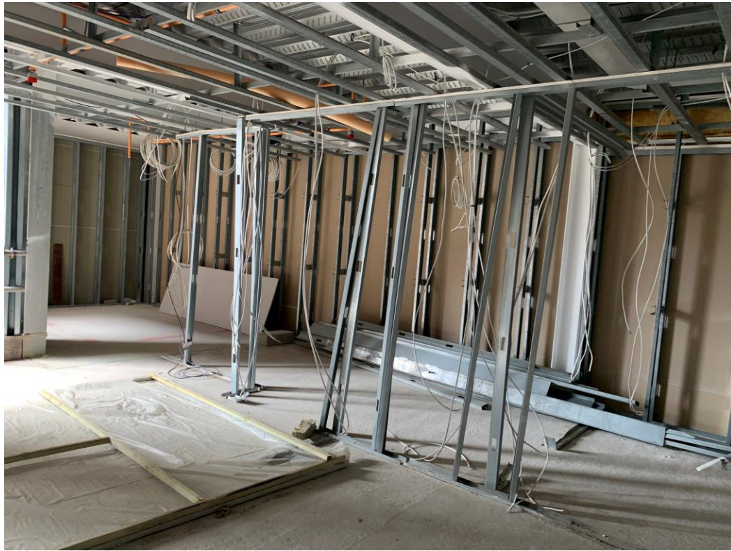
Apartment walls and ceilings under construction
