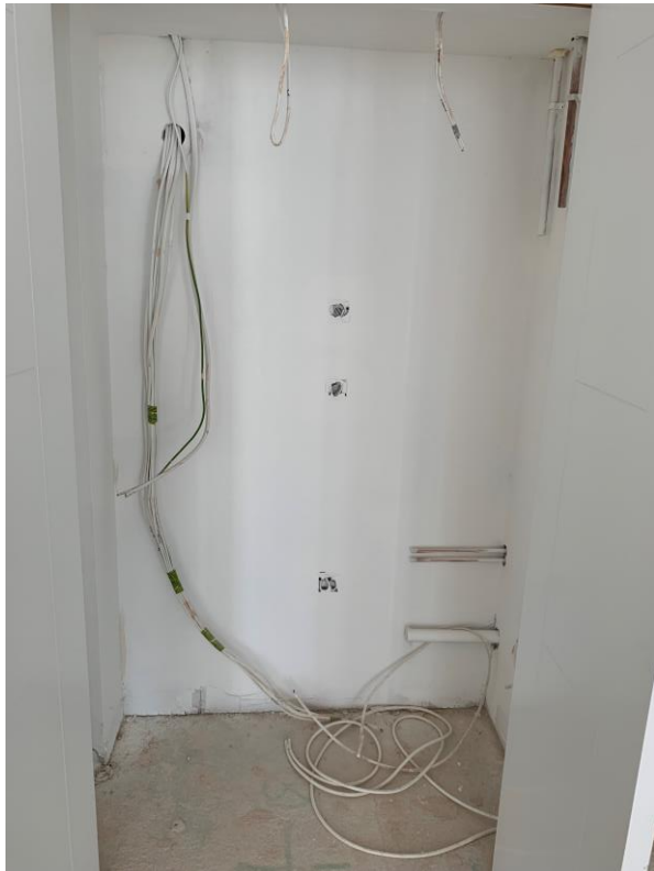
Apartment walls and ceilings mist coat /first fix electrical
