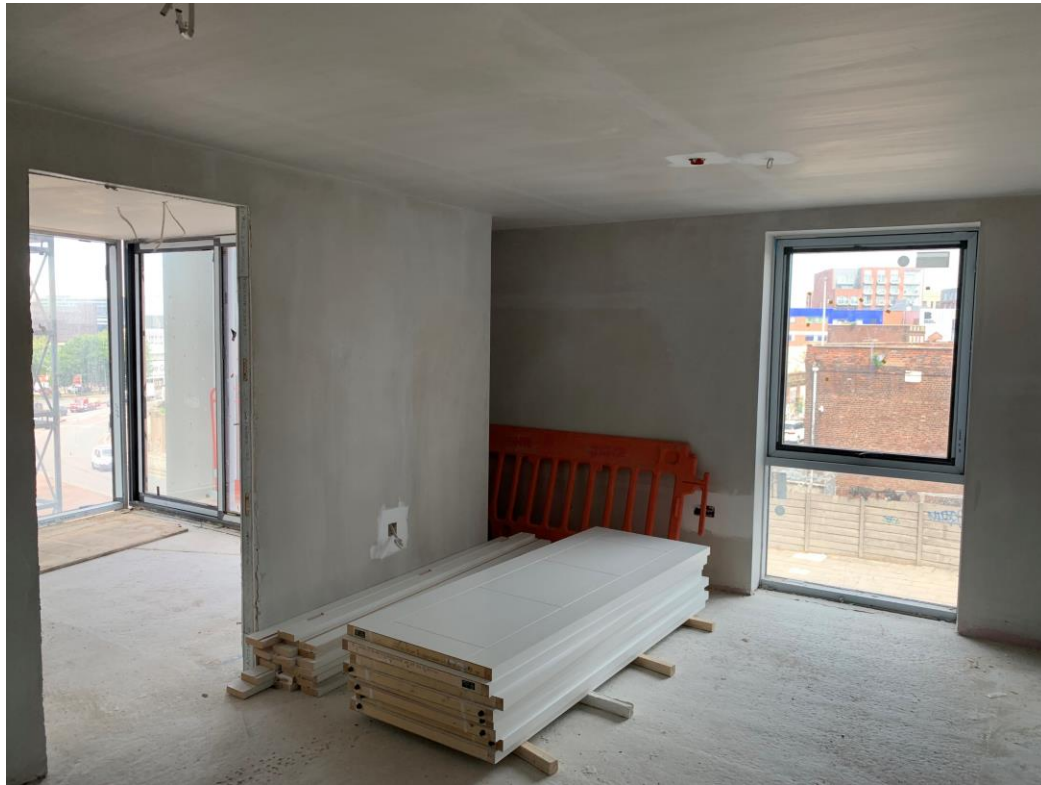
Apartment doors and frames stacked for installation
