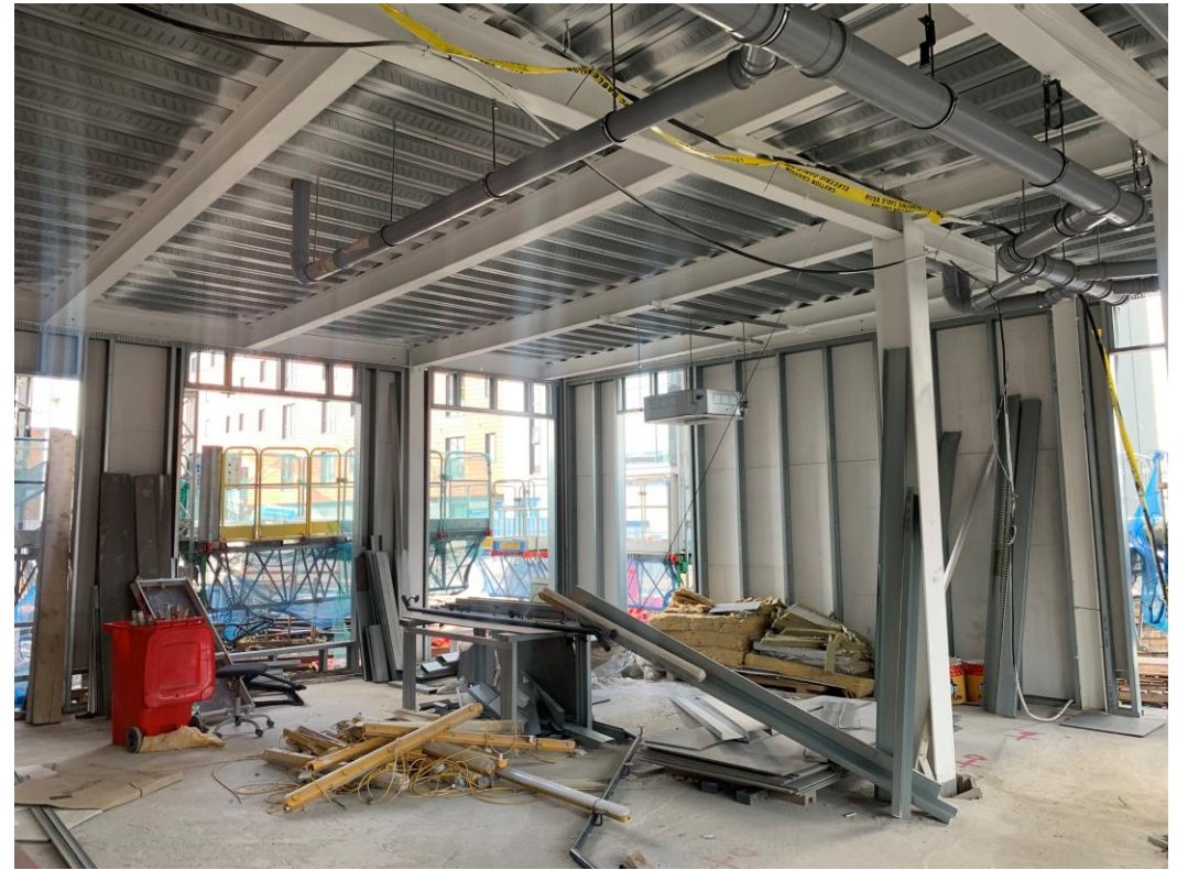
Ground Floor walls and ceilings under construction /above ground drainage
