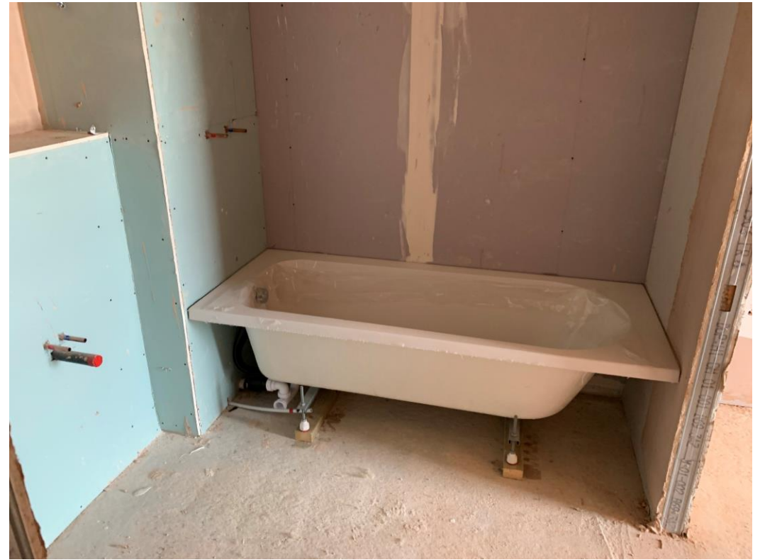
Apartment sanitary first fix
