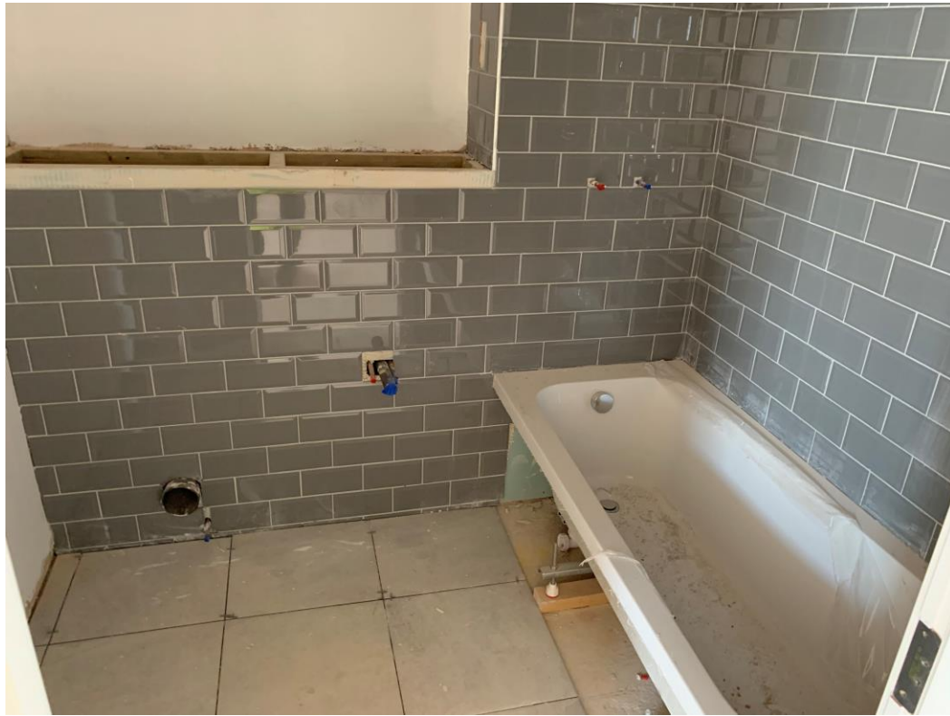
Bathroom wall and floor tiling commenced
