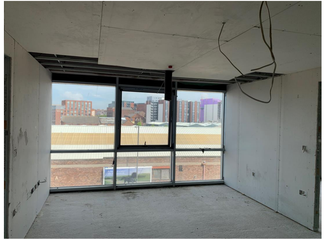
Apartment walls and ceilings boarded
