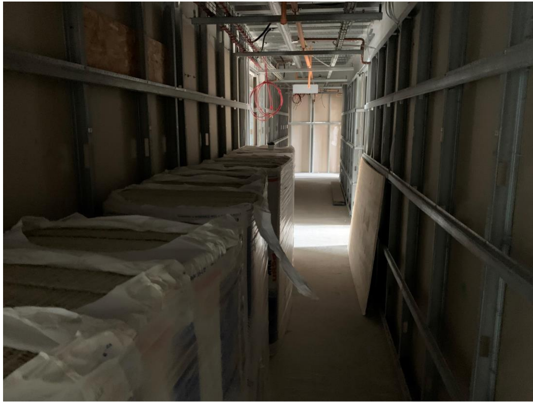
Corridor walls and ceilings under construction
