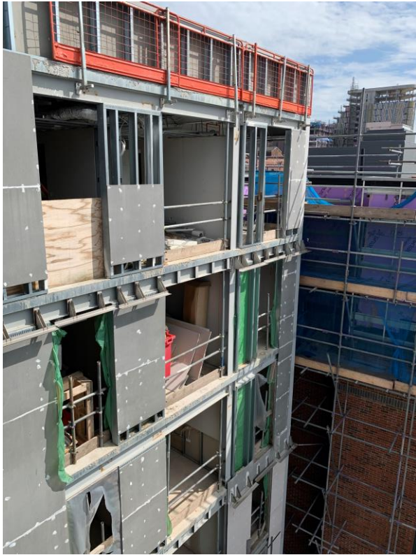
External cladding under construction
