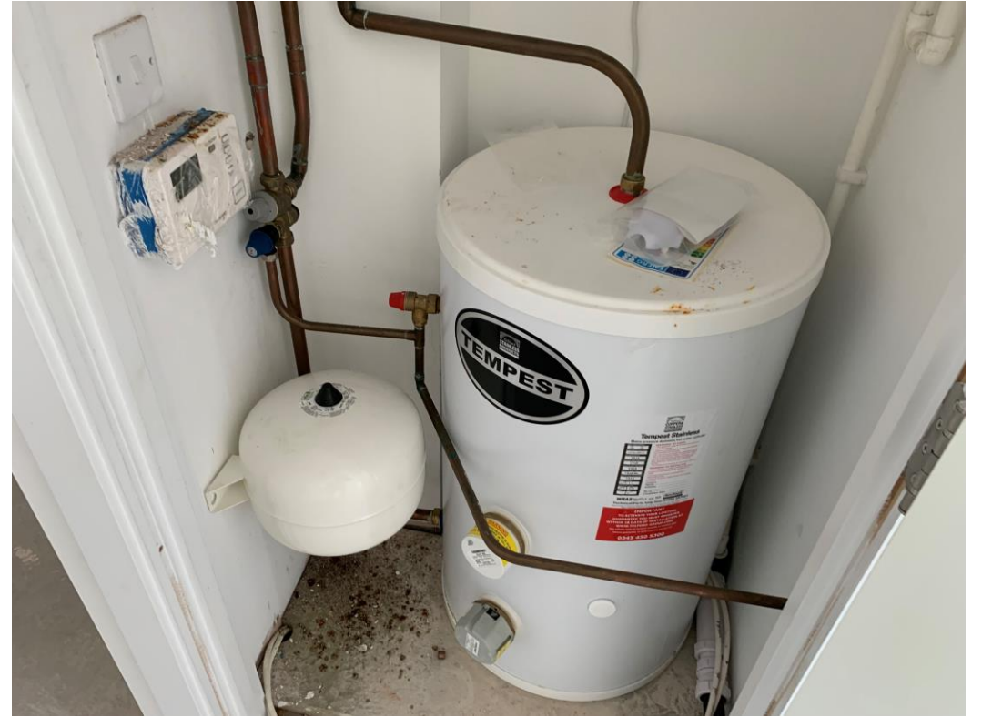
Water cylinder installed
