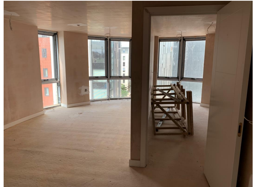
Apartment plaster skimmed /second fix joinery
