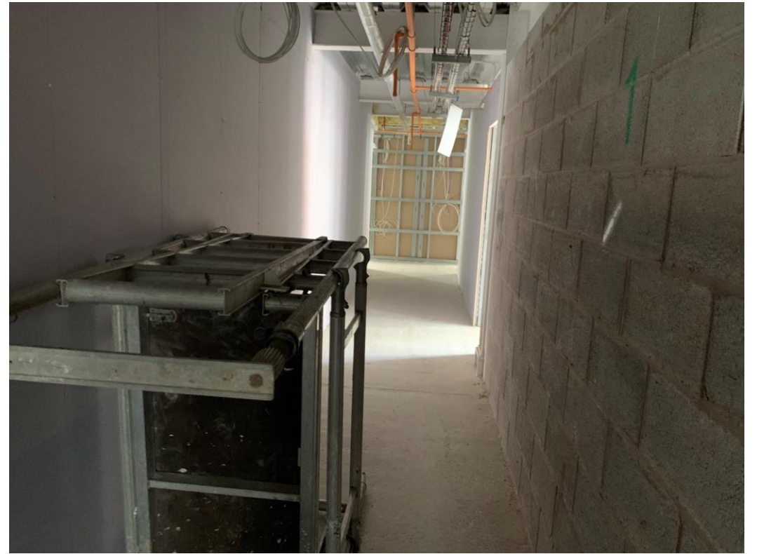
Corridor walls and ceilings under construction
