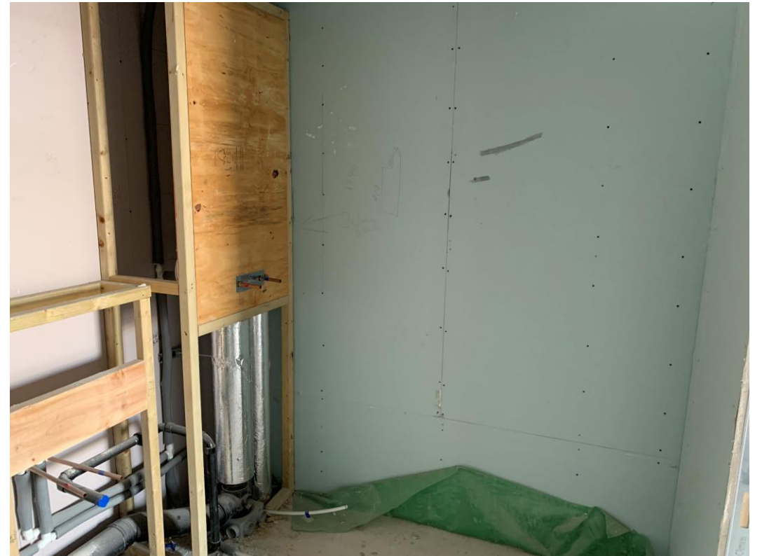
Apartment walls and ceilings under construction
