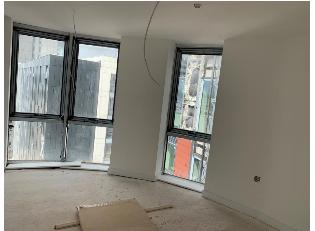
Apartment walls and ceilings mist coat /first fix electrical
