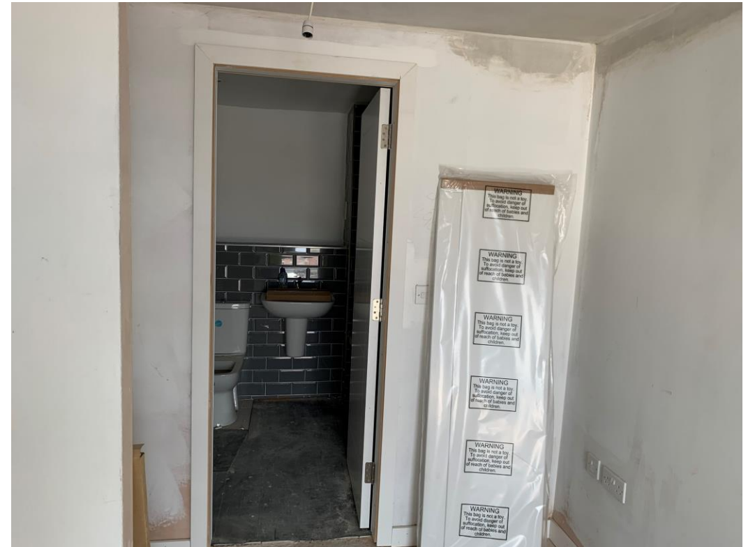
Apartment doors and frames installed
