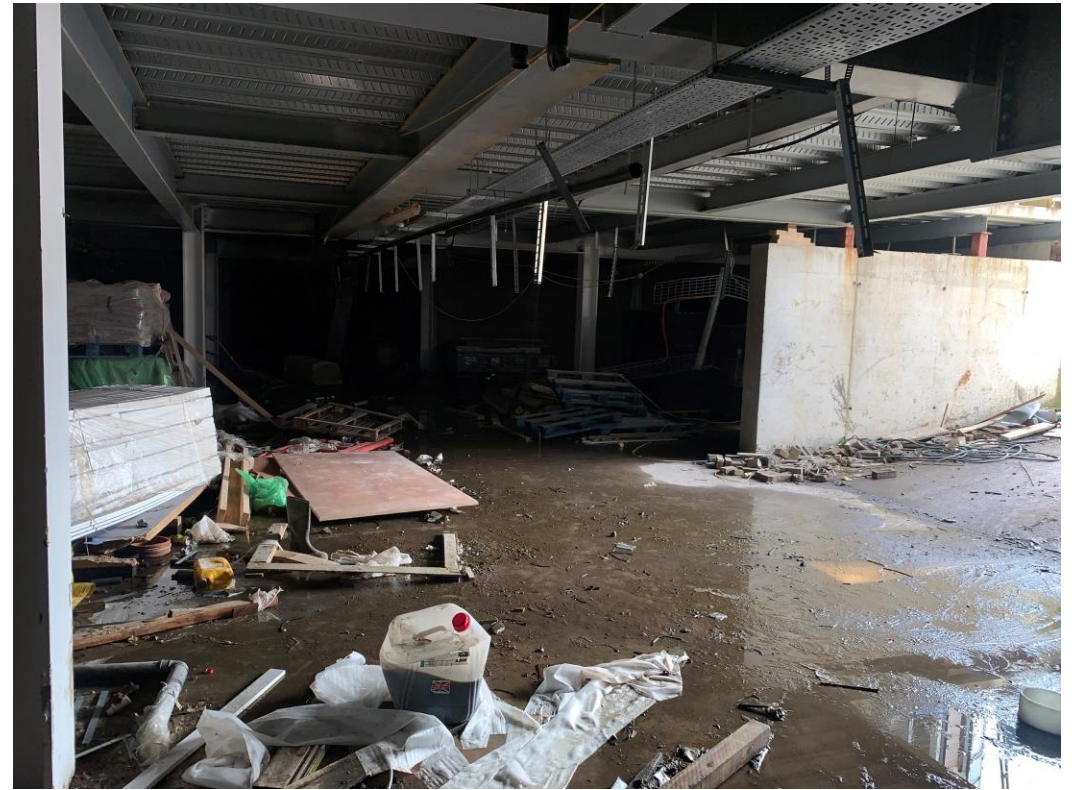
Basement ramp access
