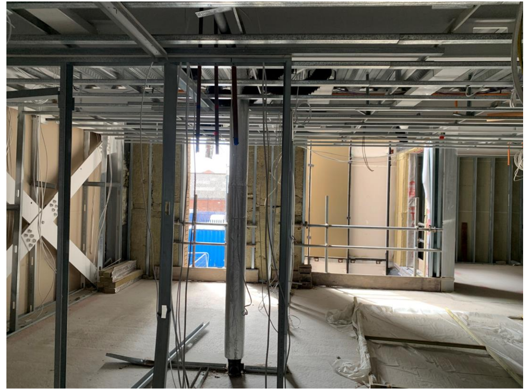
Apartment walls and ceilings under construction
