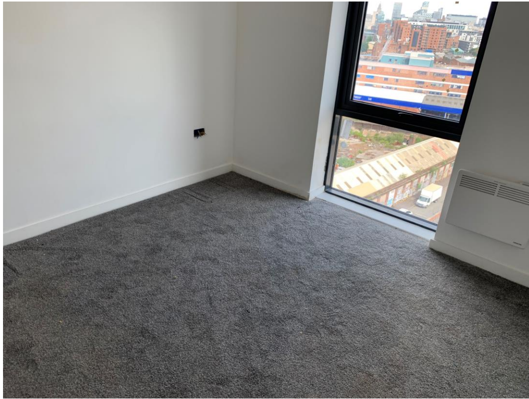
Apartment fitout advanced
