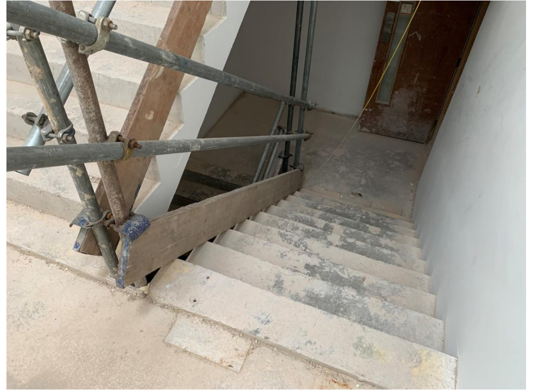
Tenth Floor stairwell
