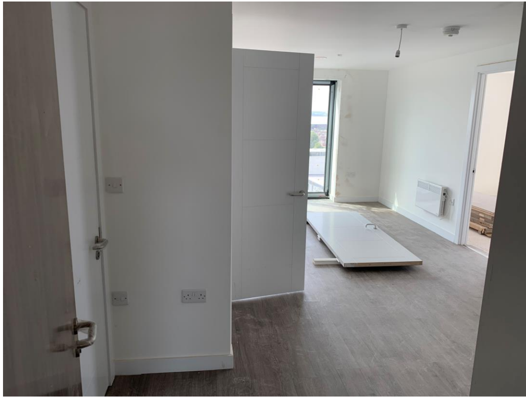
Apartment fitout advanced
