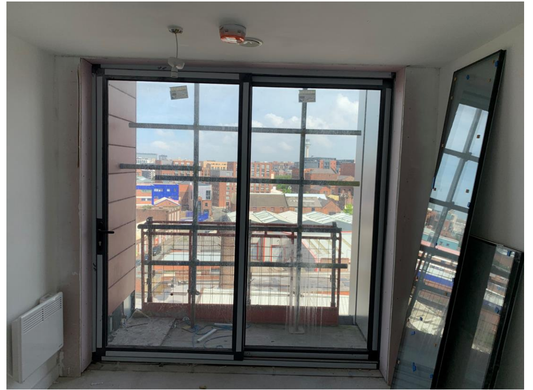
Apartment balcony doors
