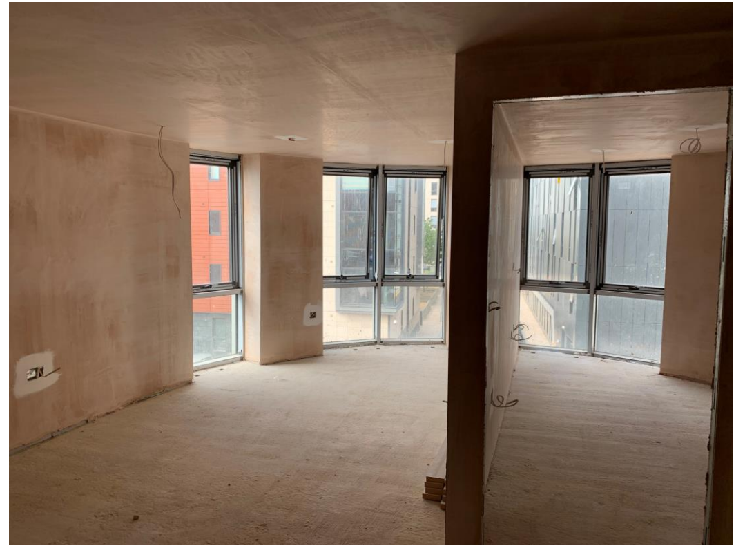
Apartment walls and ceilings under construction
