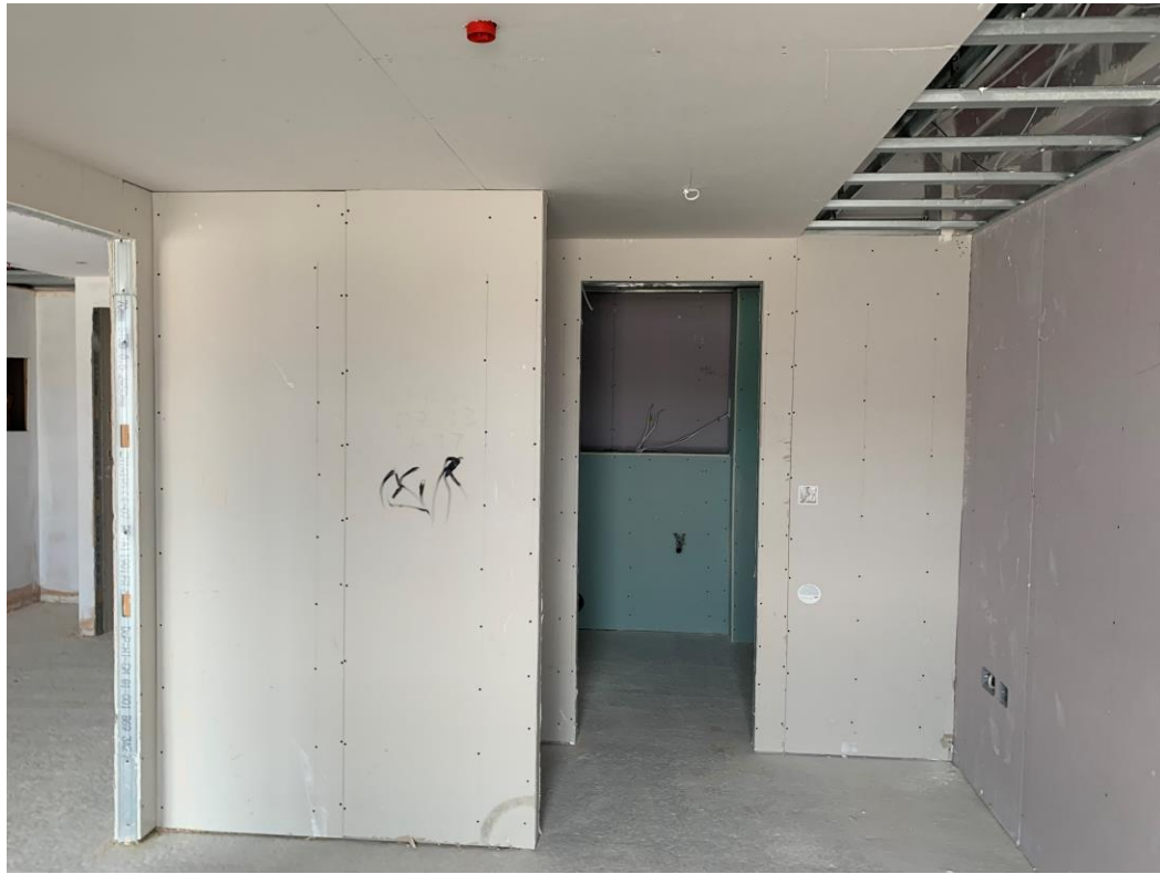
Apartment walls and ceilings boarded
