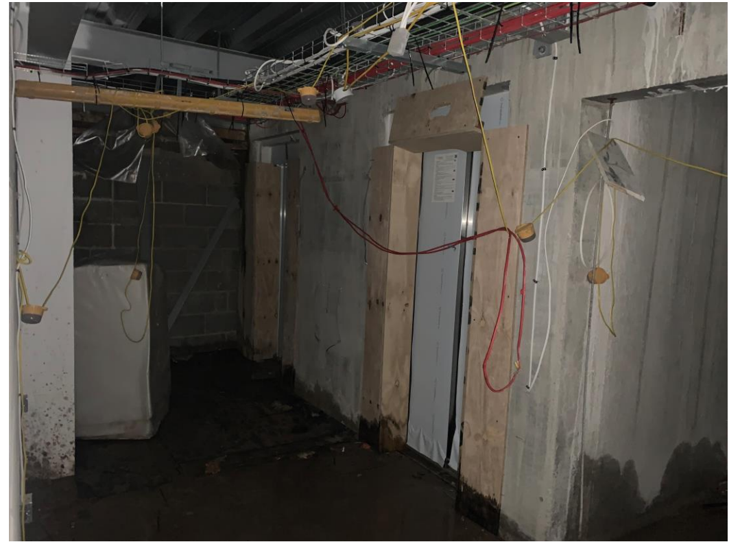
Basement lift access
