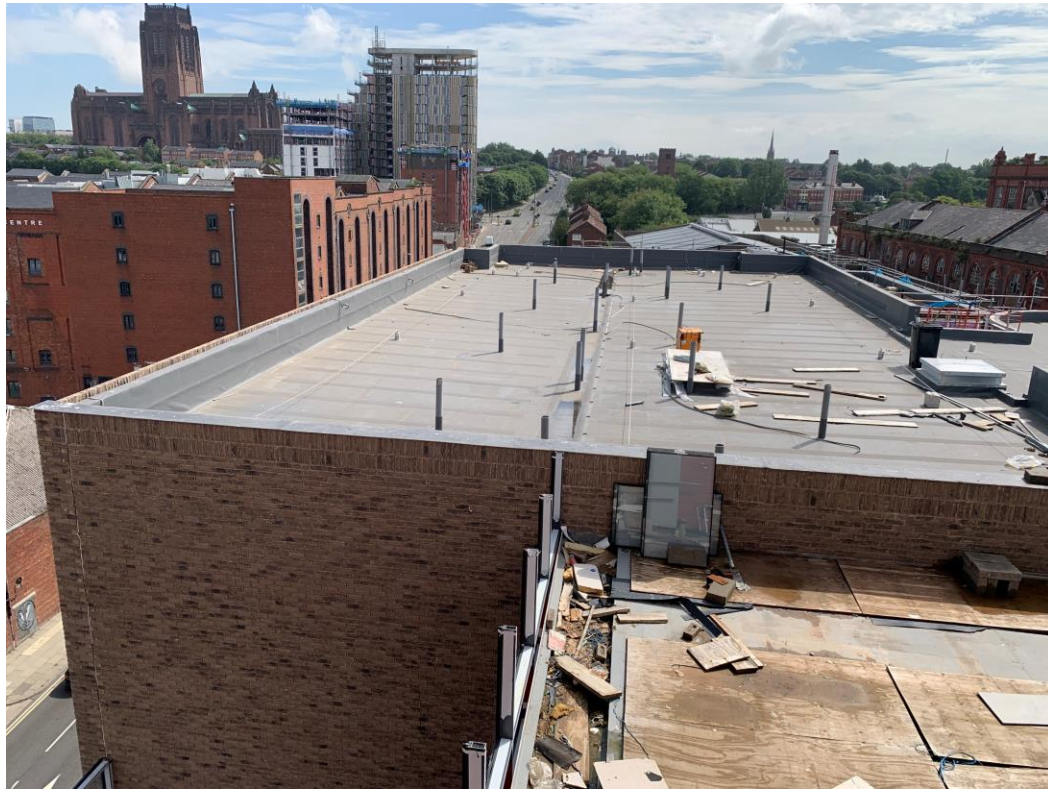
Main flat roof covering
