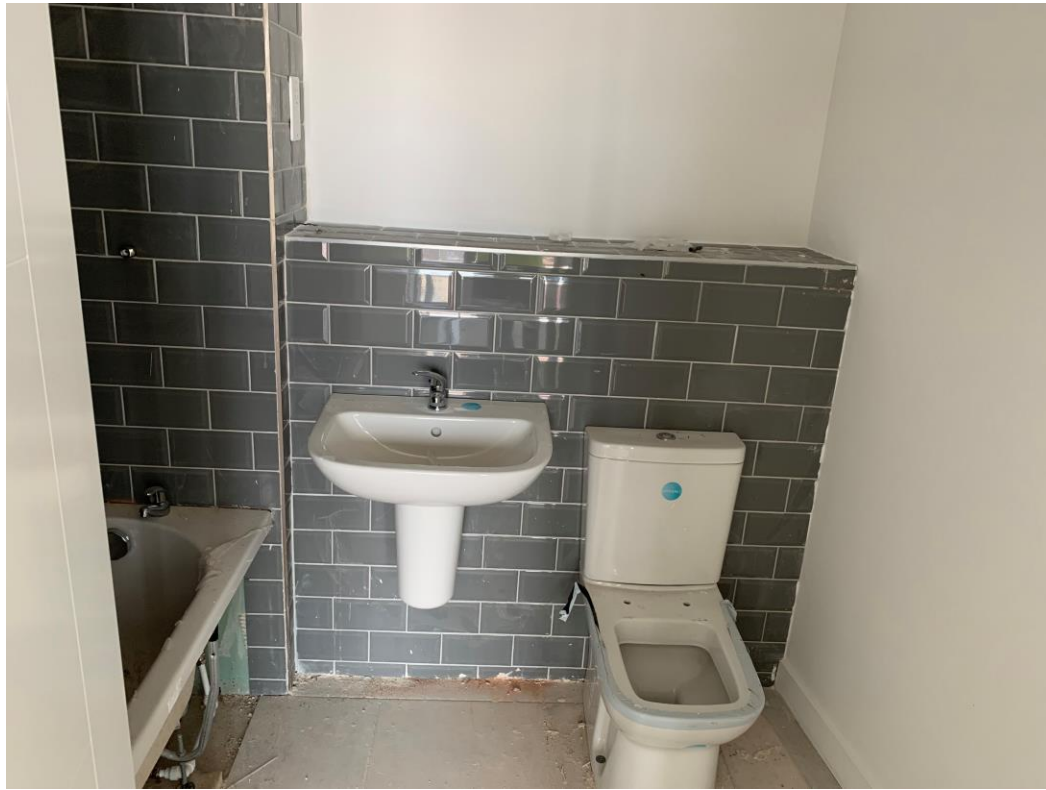
Bathroom sanitary fittings commenced
