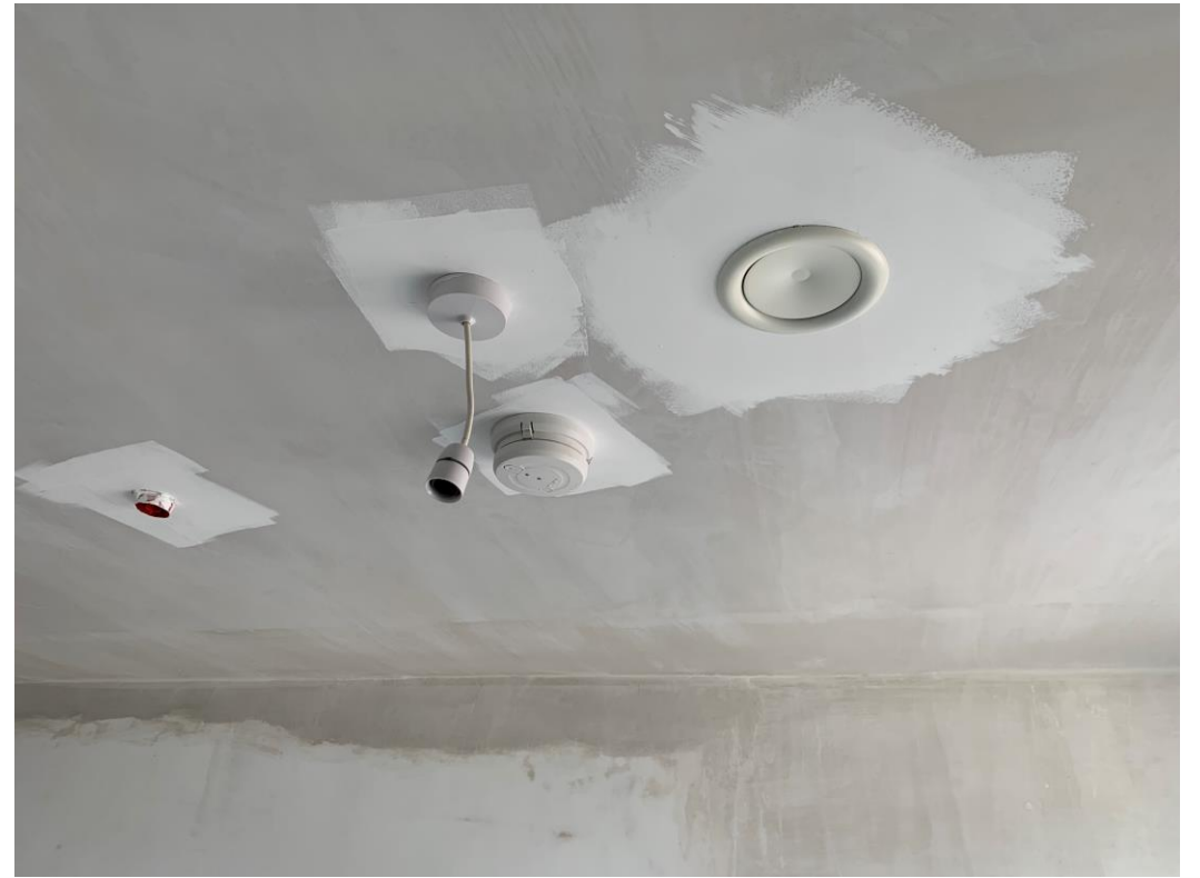
Apartment second fix mechanical and electrical
