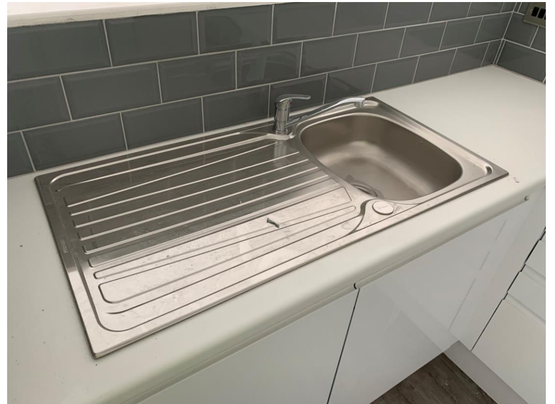
Apartment fitout advanced
