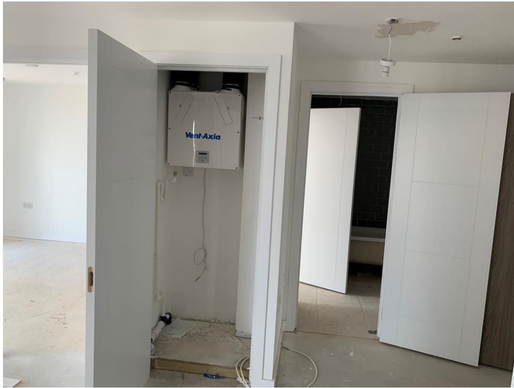
Apartment doors and frames installed
