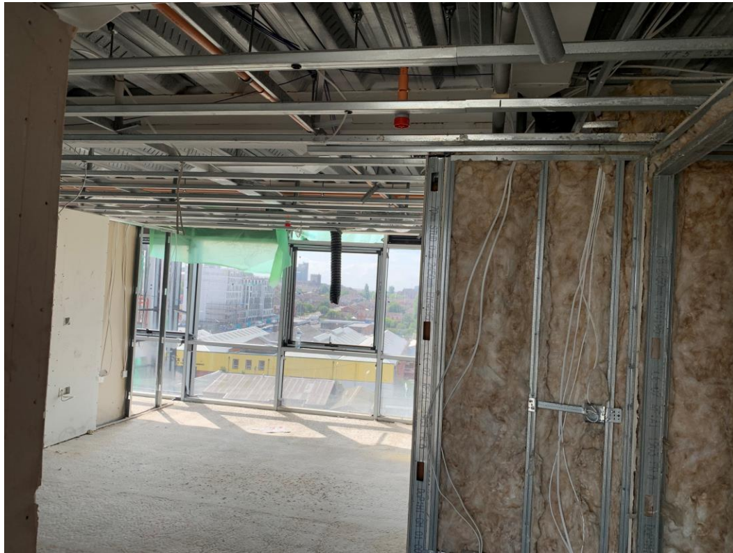
Apartment walls and ceilings under construction
