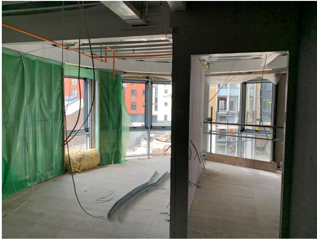
Apartment walls and ceilings under construction
