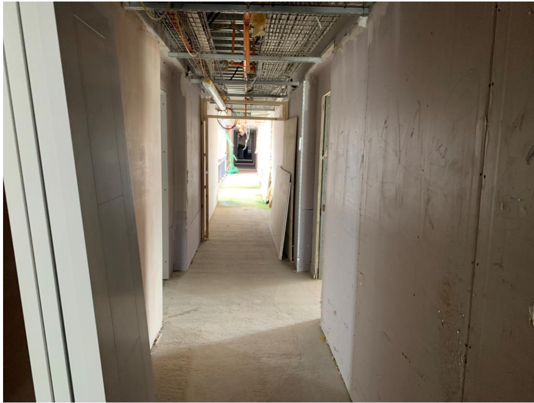
Corridor walls and ceilings under construction
