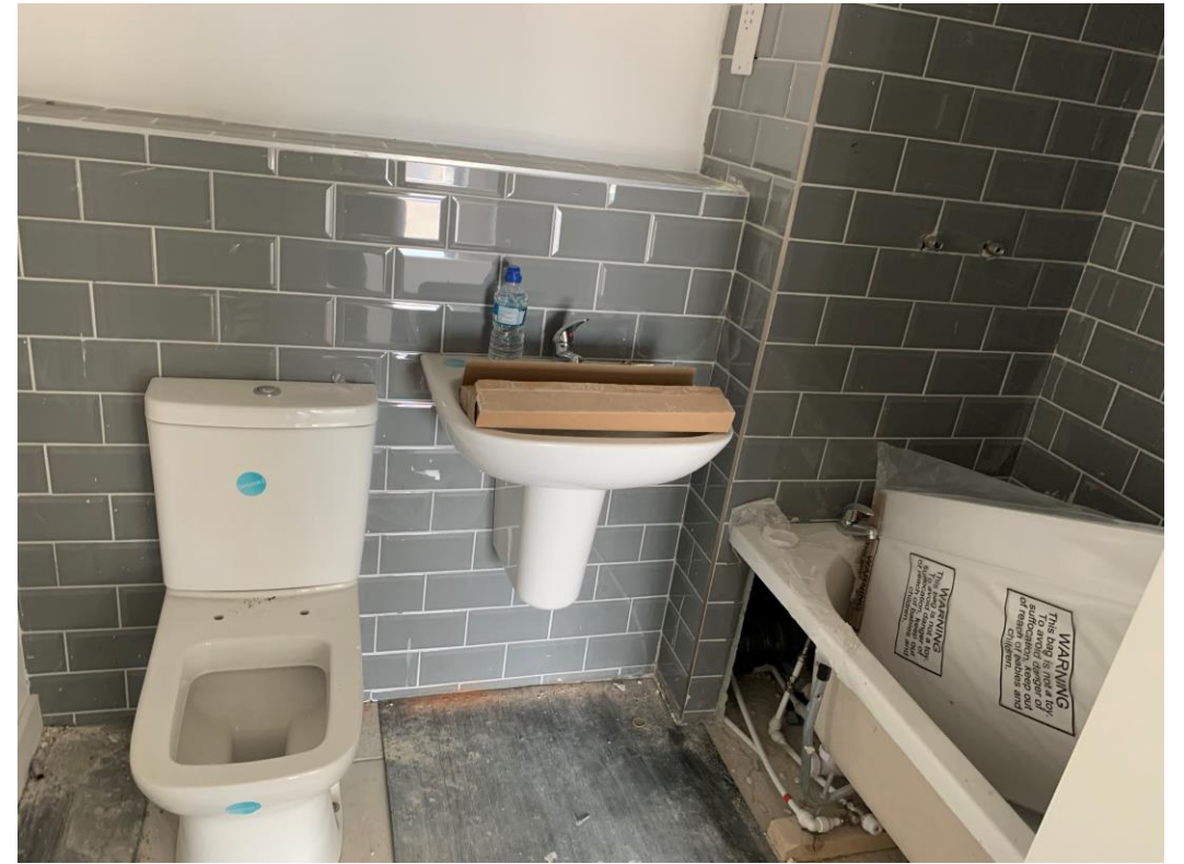
Bathroom sanitary fittings commenced
