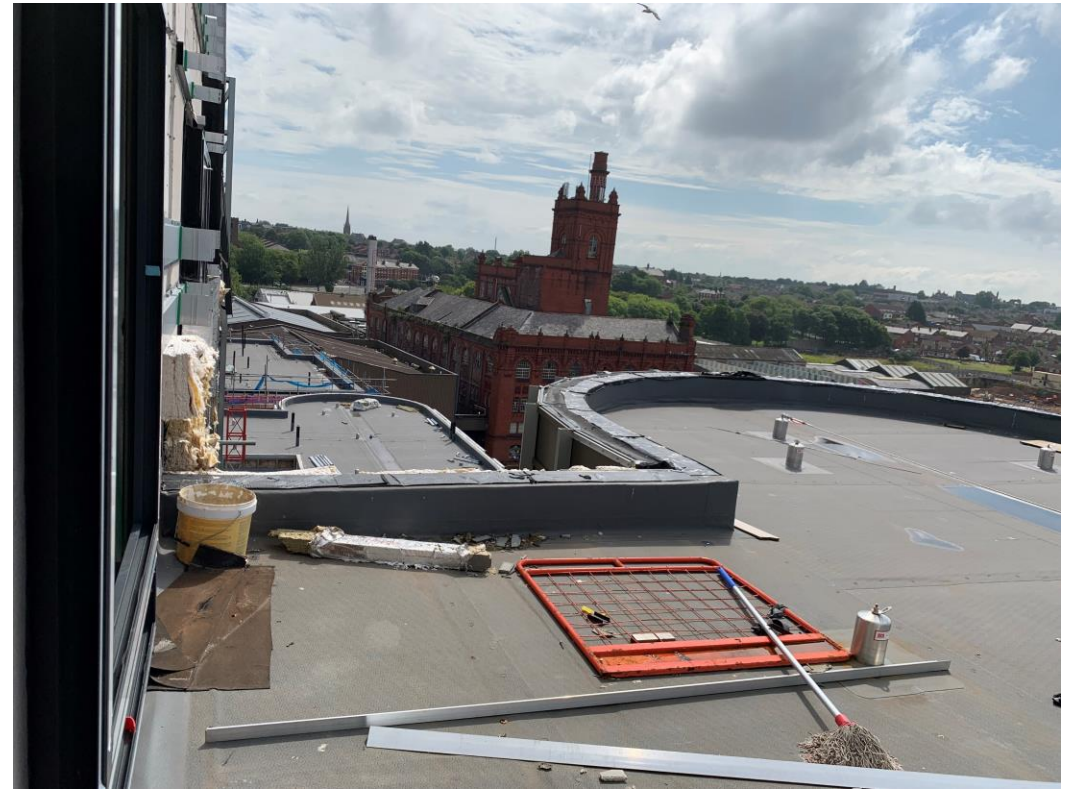
Main flat roof covering
