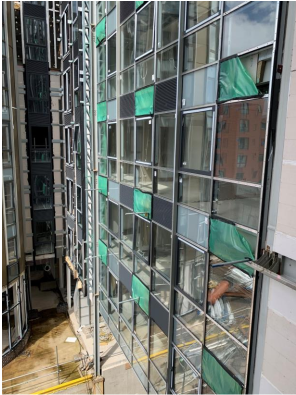
Curtain walling and windows installed
