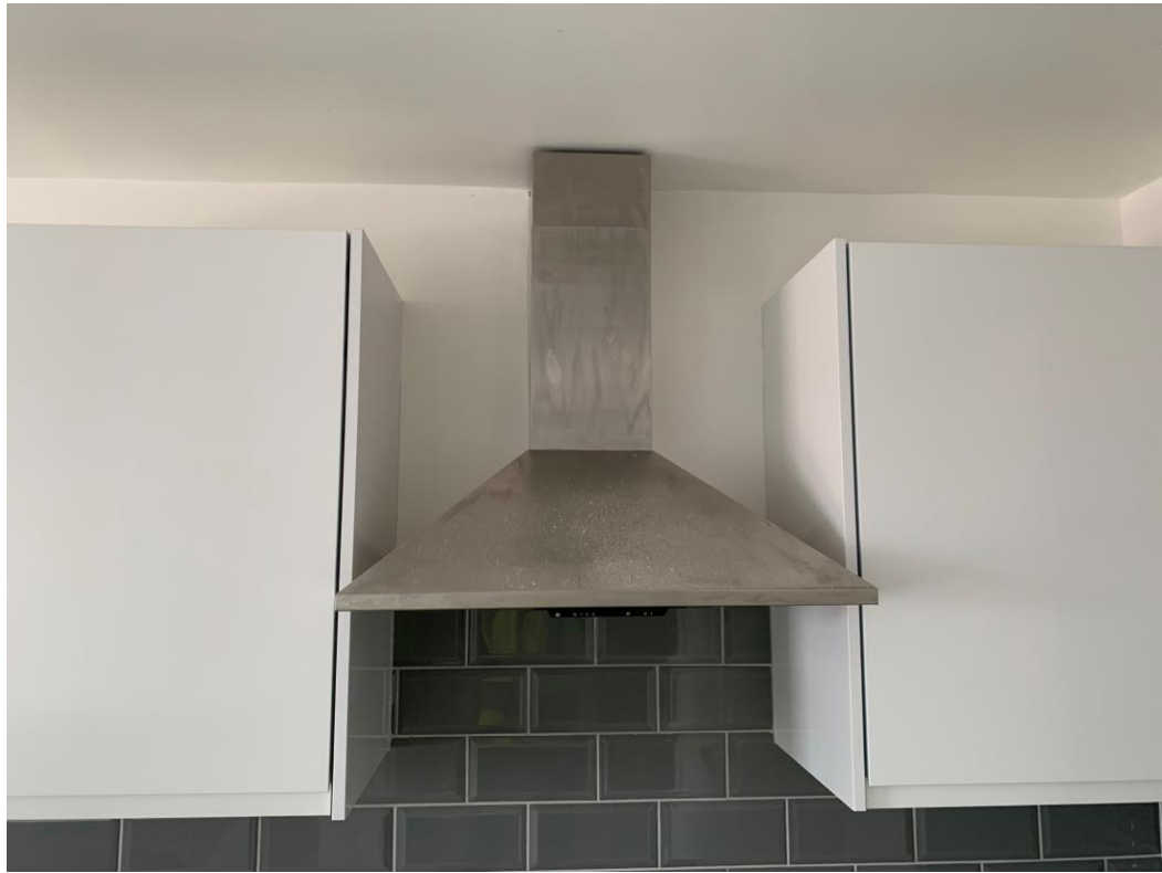
Apartment fitout advanced
