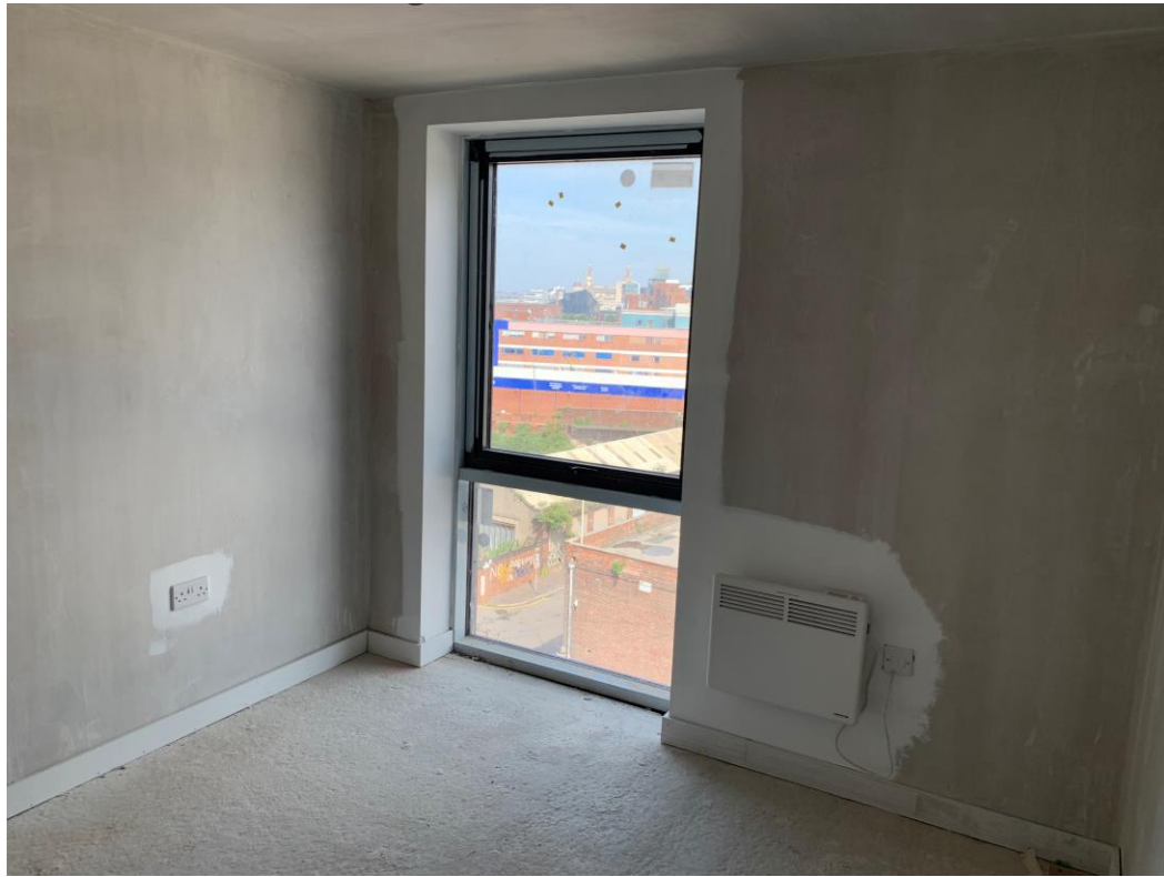
Apartment second fix mechanical and electrical
