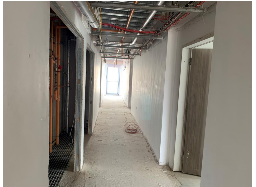
Corridor walls and ceilings under construction
