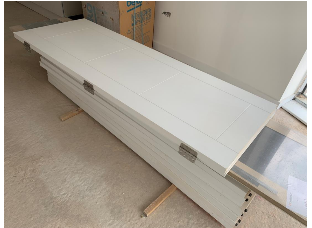
Apartment doors stacked for installation
