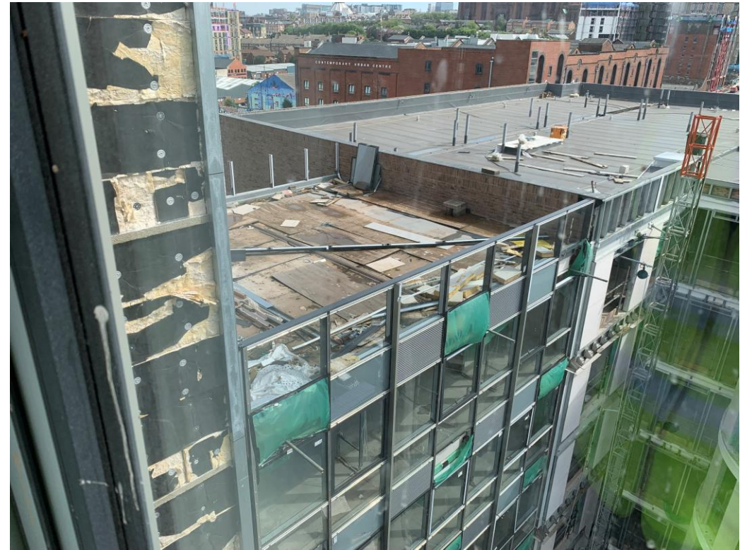
Main flat roof covering and terrace
