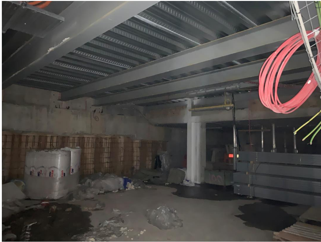
Basement steel framework
