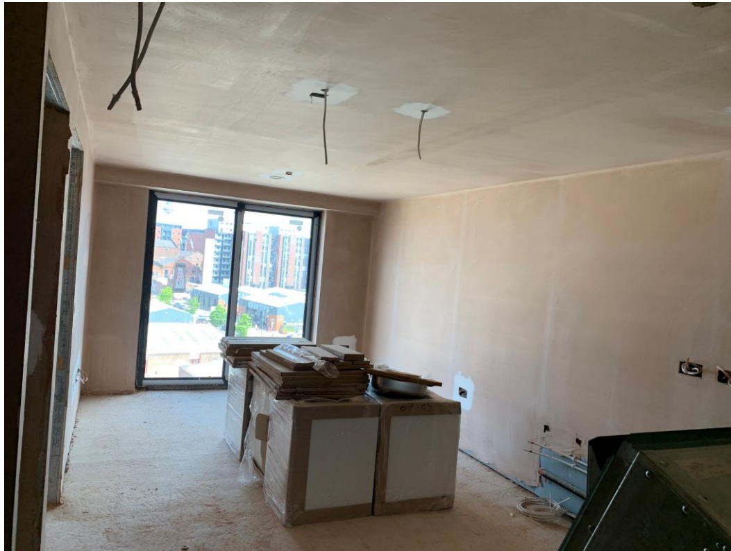
Apartment plumbing & electrical first fix
