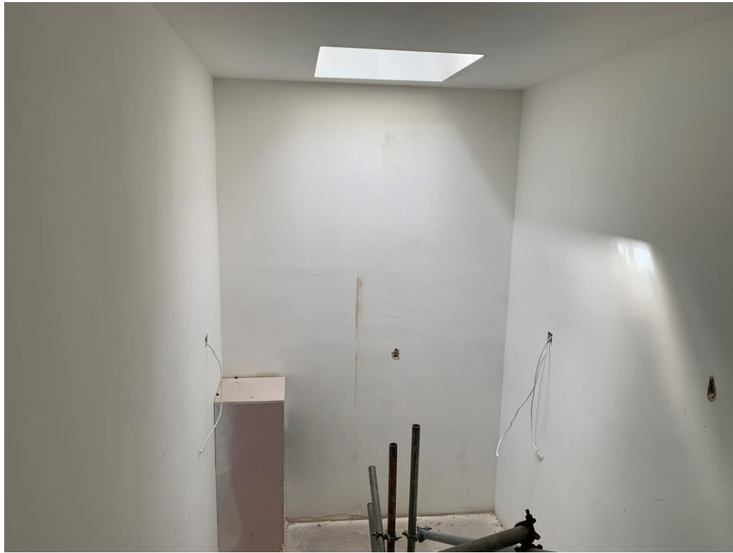
Tenth Floor stairwell
