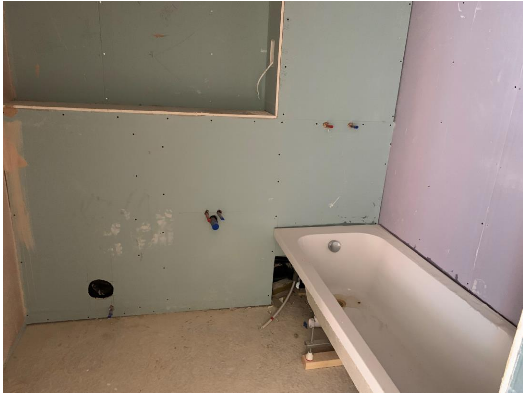
Apartment sanitary first fix
