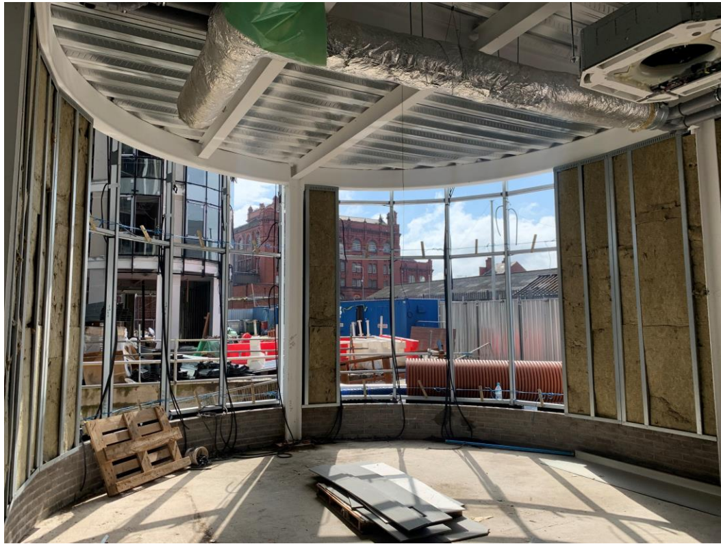
Ground Floor walls and ceilings under construction /mechanical plant
