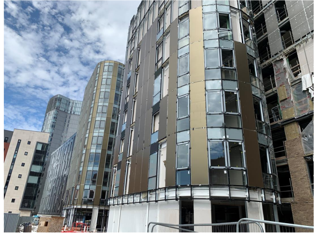
Development viewed from Brindley Street
