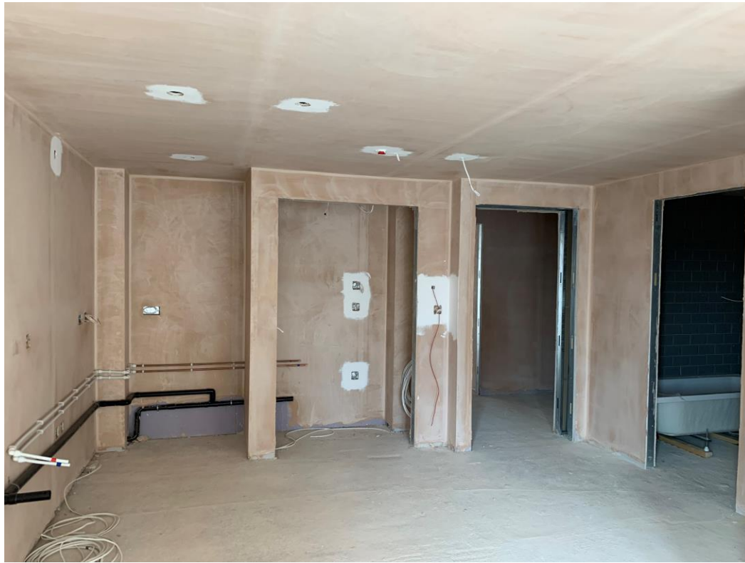
Apartment plumbing first fix
