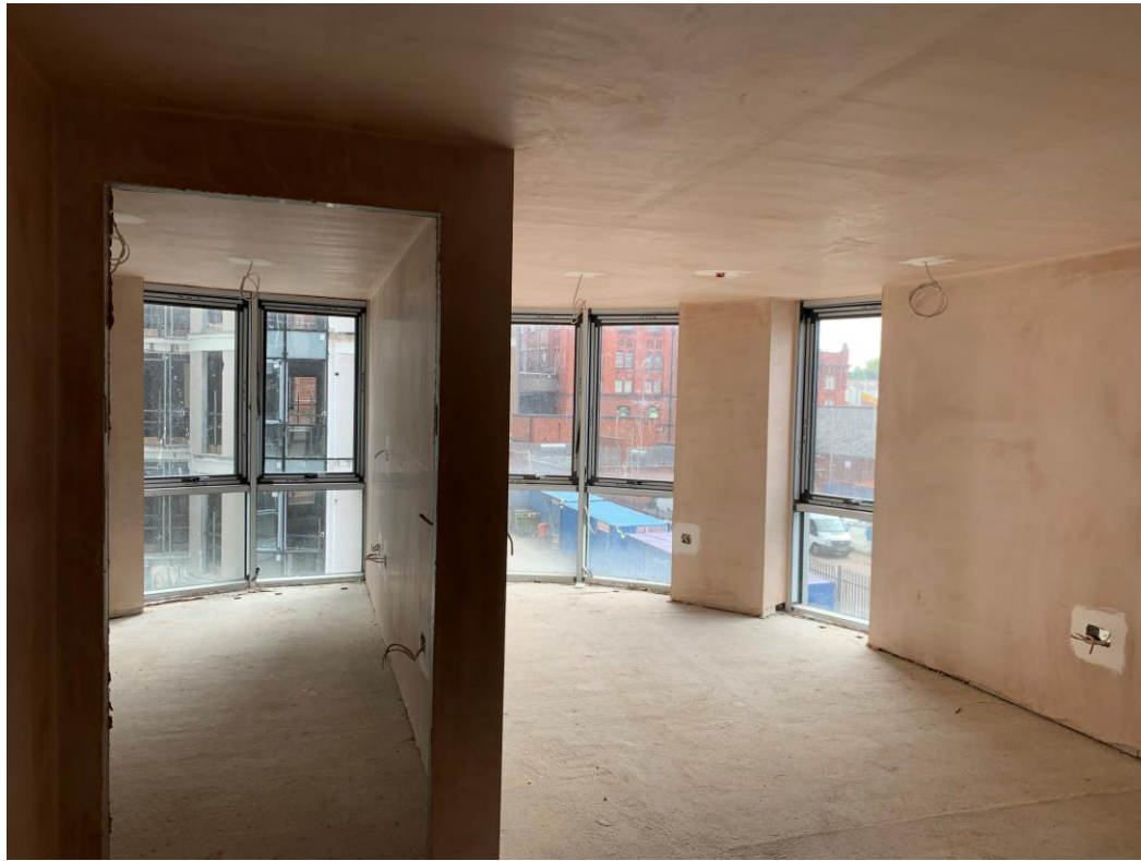
Apartment plaster skimmed
