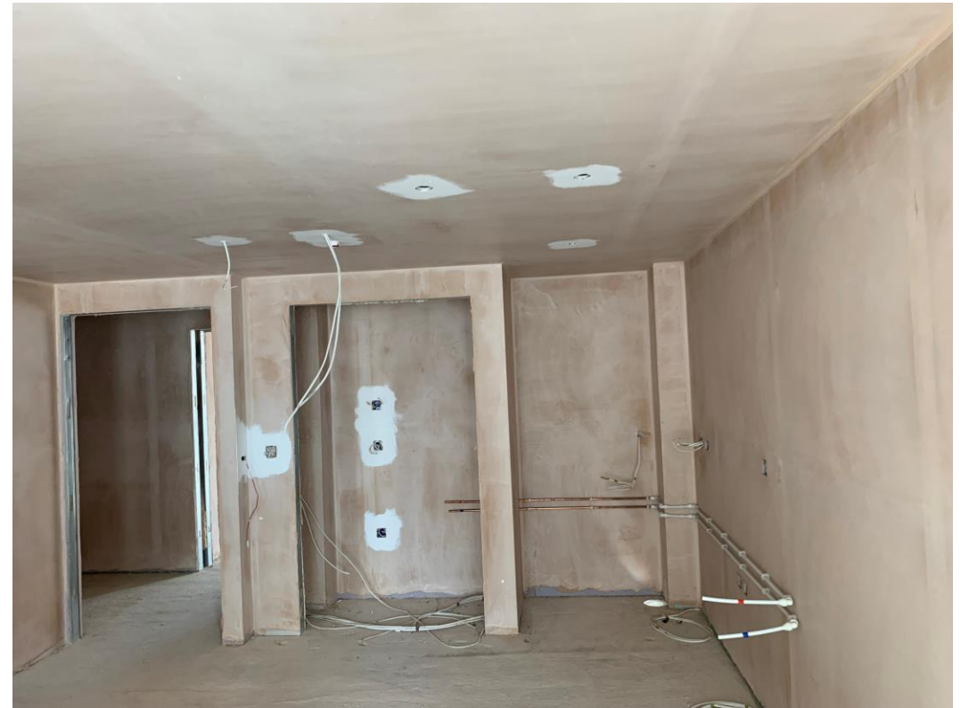
Apartment plumbing & electrical first fix
