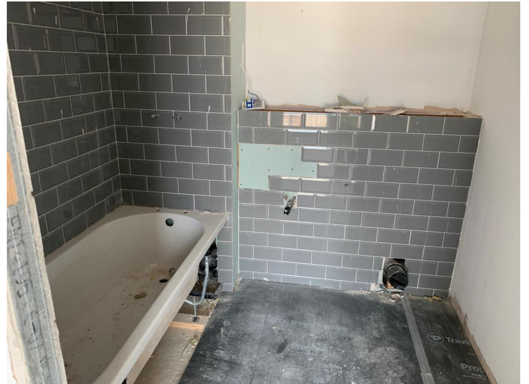
Bathroom wall and floor tiling commenced
