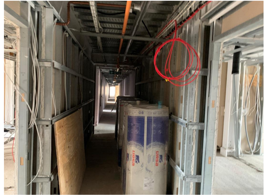
Corridor walls and ceilings under construction
