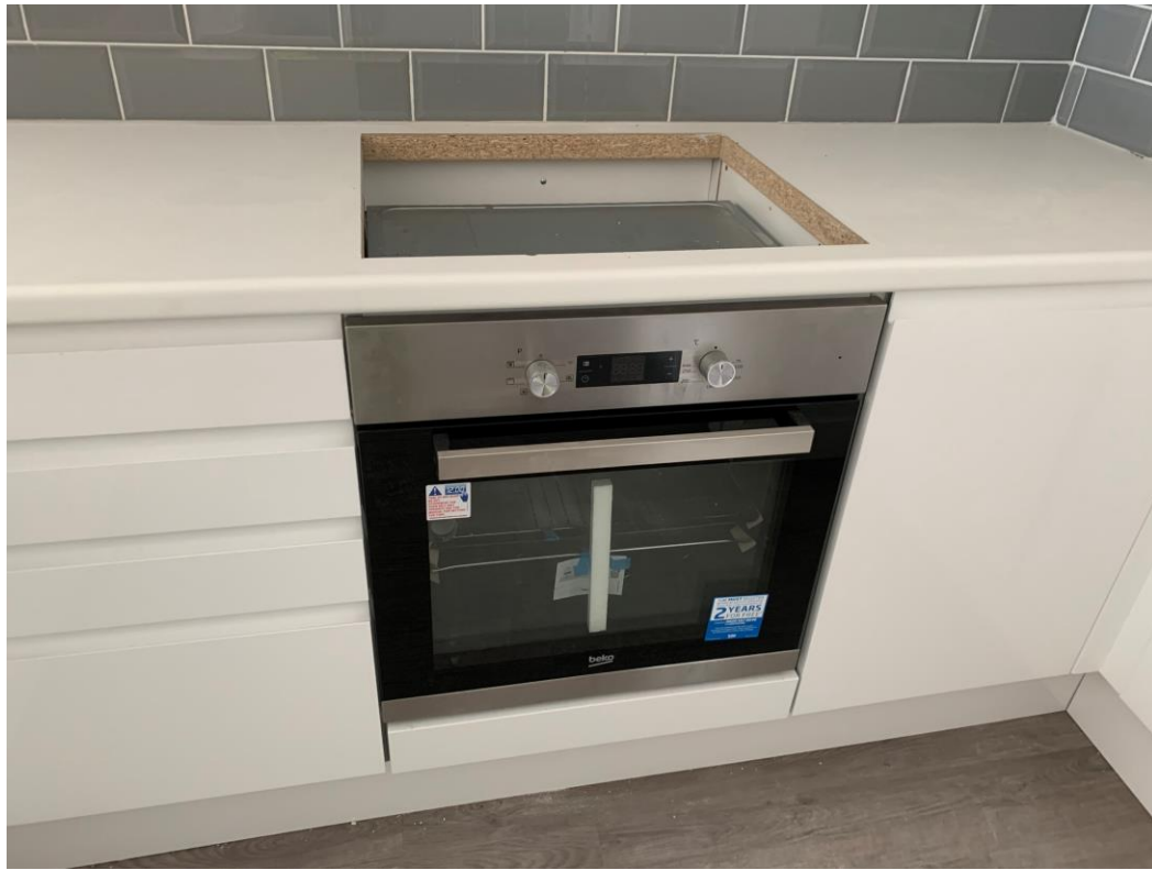
Apartment fitout advanced
