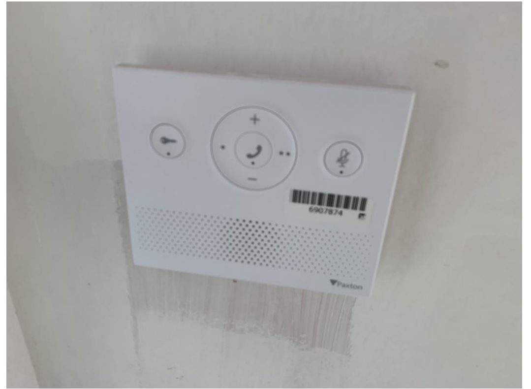
Apartment fitout advanced
