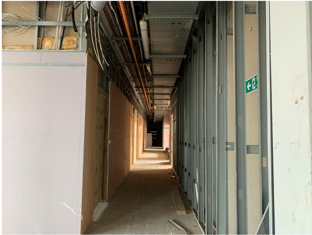
Ground Floor walls and ceilings under construction /electrical services
