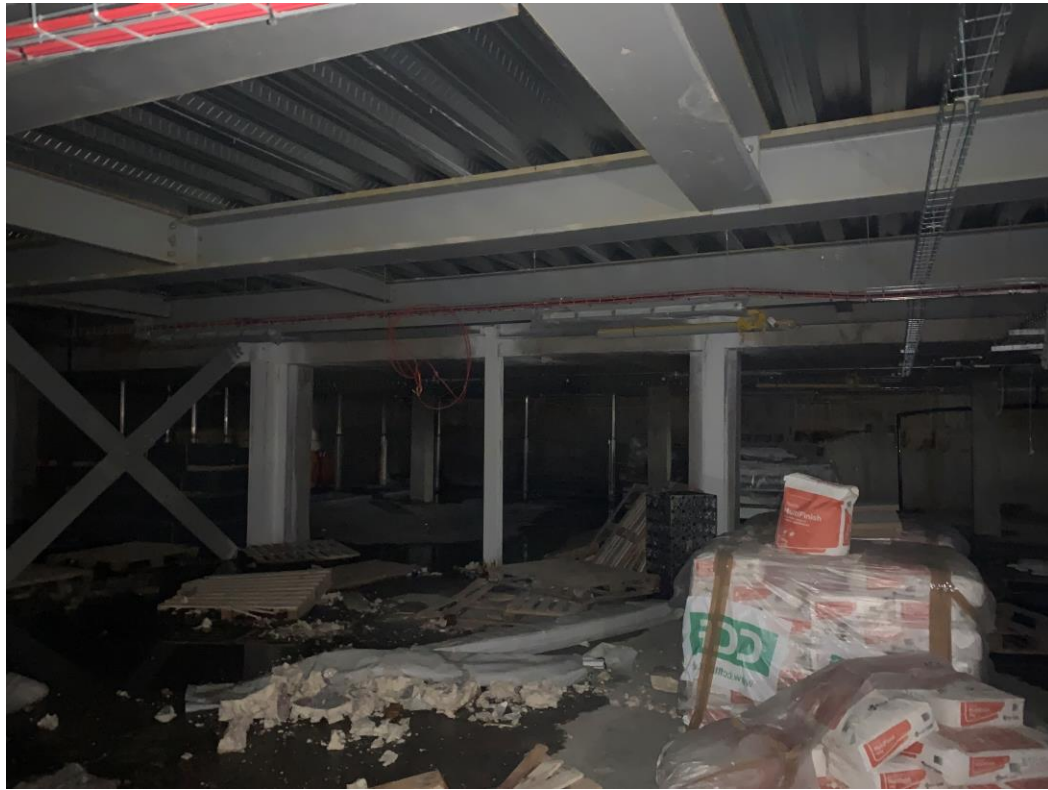
Basement steel framework
