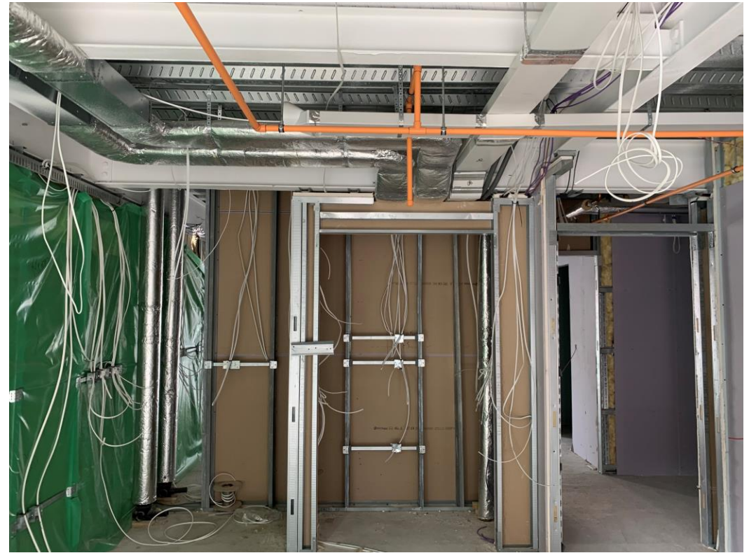
Apartment walls and ceilings under construction
