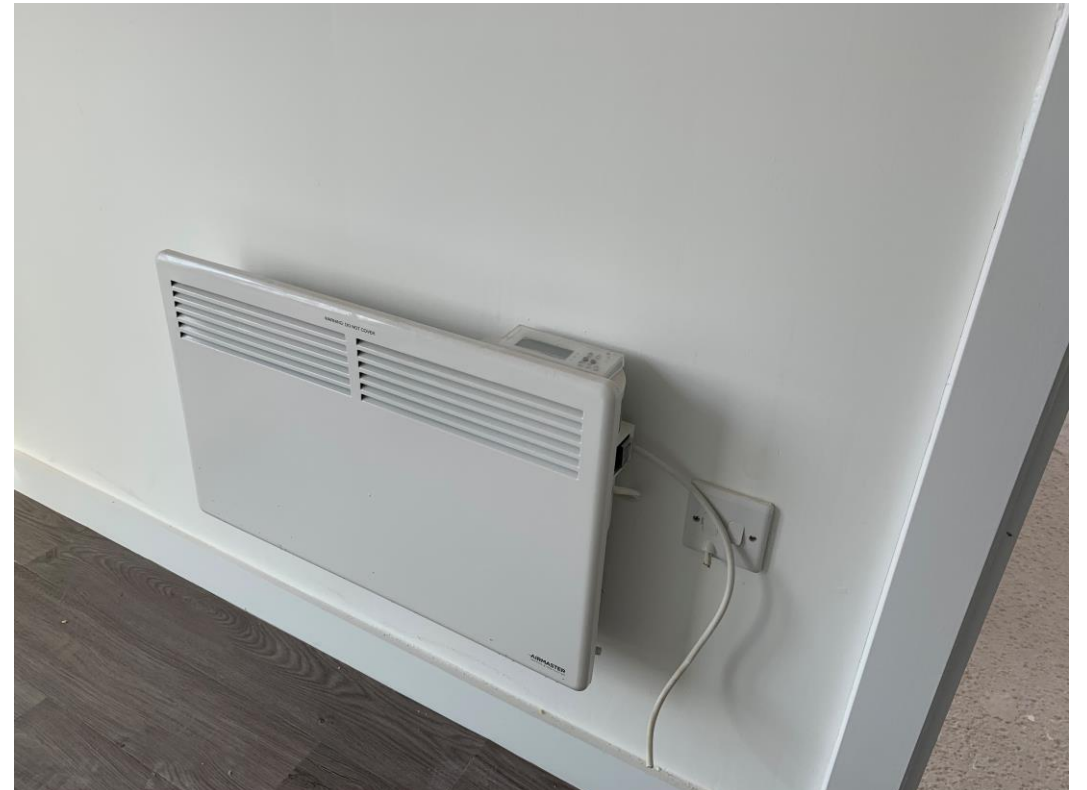
Apartment fitout advanced
