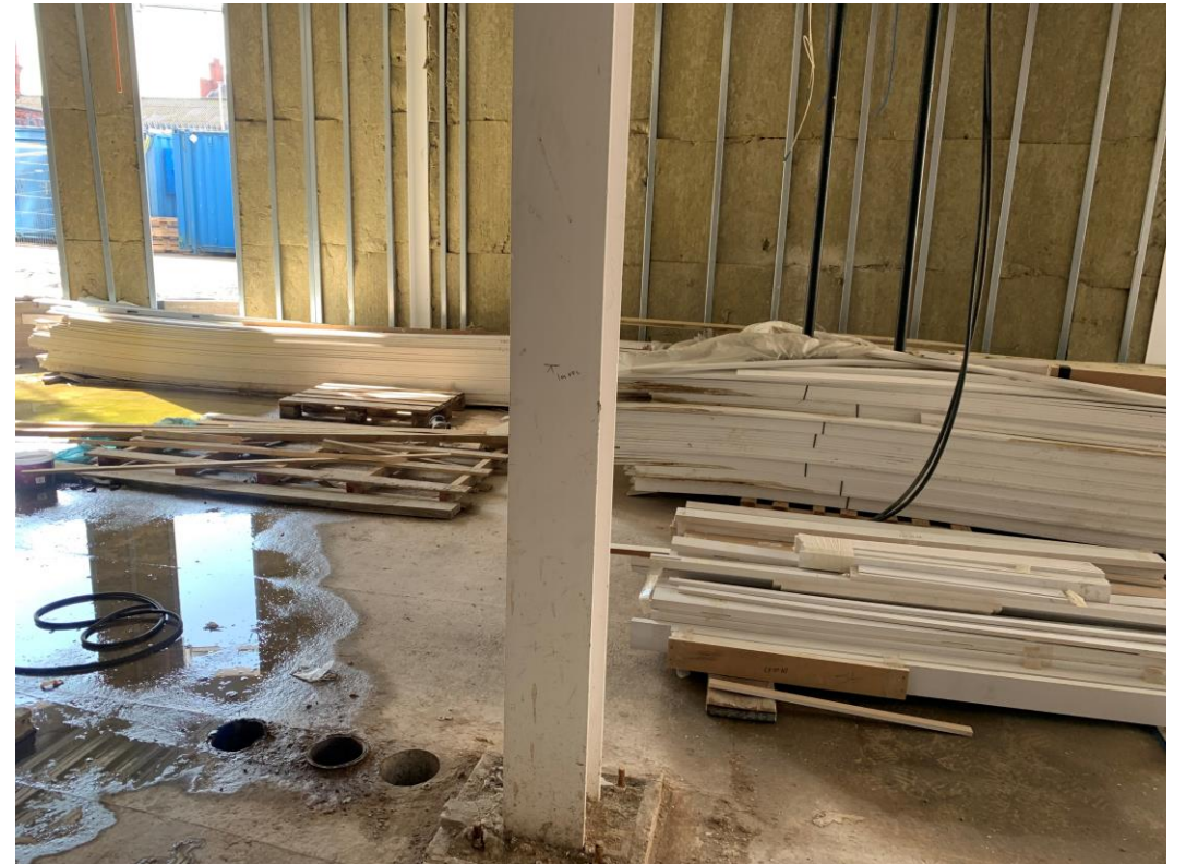
Ground Floor core drill holes
