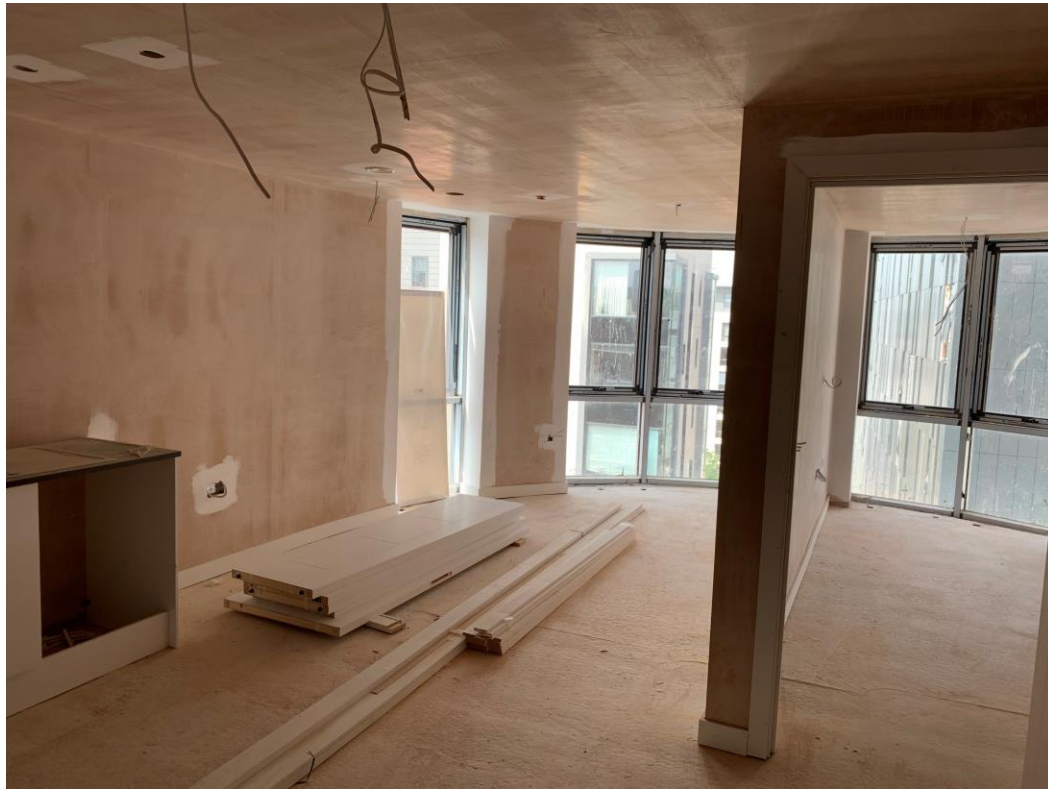
Apartment plaster skimmed /second fix joinery
