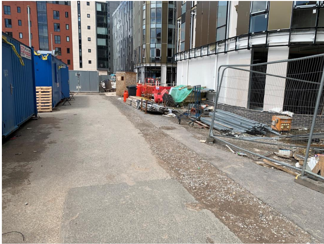
Development access road viewed from Caryl Street
