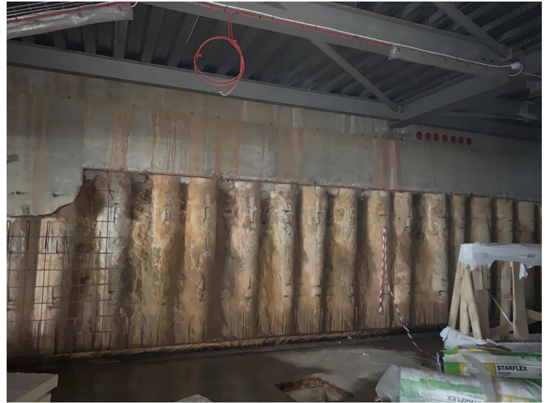
Basement wall structure
