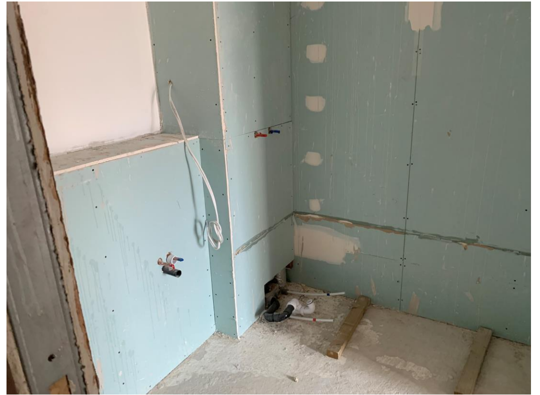
Apartment walls and ceilings under construction
