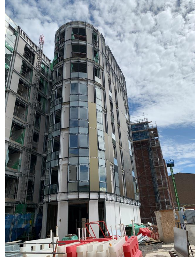
Development viewed from Brindley Street
