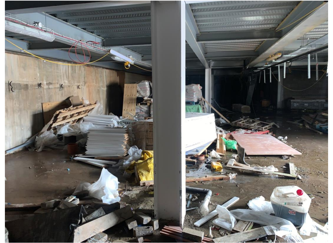
Basement steel framework
