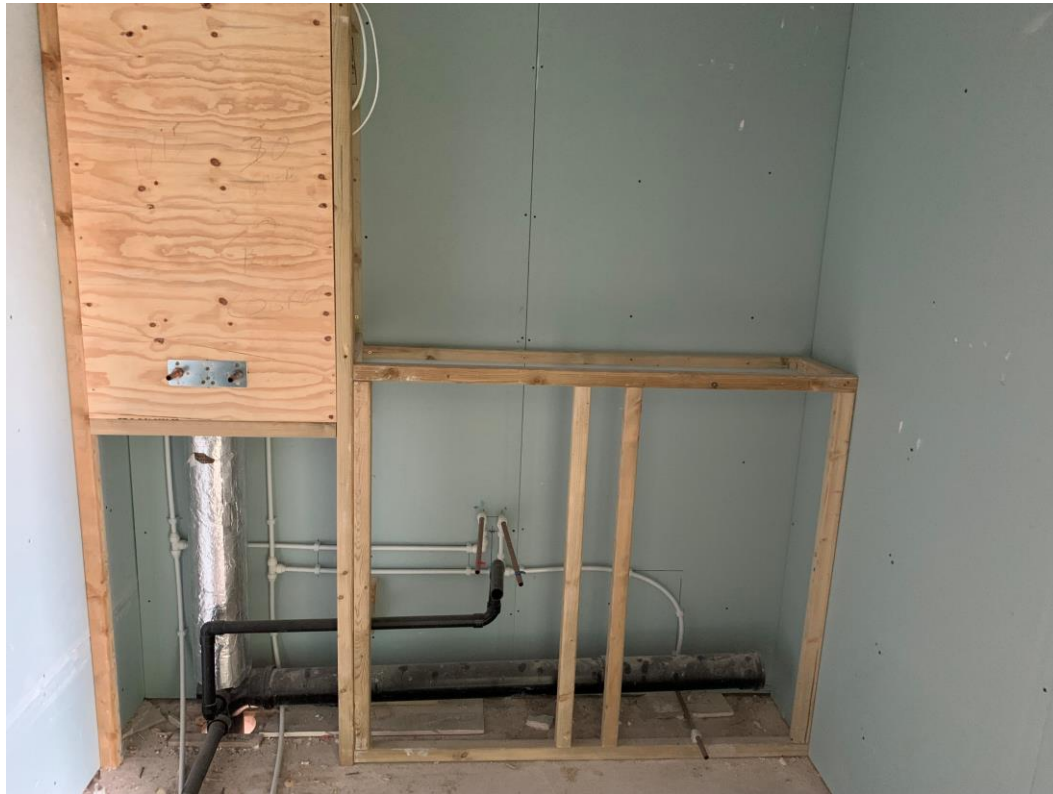
Apartment Bathroom IPS under construction
