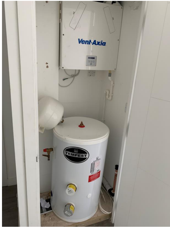
Mechanical ventilation & water cylinder installed
