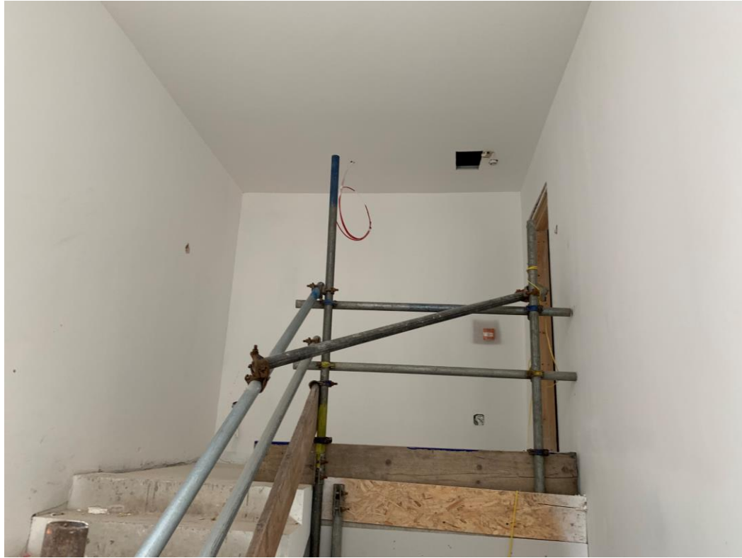
Tenth Floor stairwell
