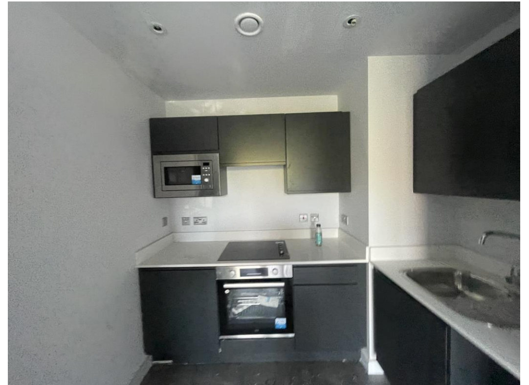
Level 3 – kitchen units & worktops installed
