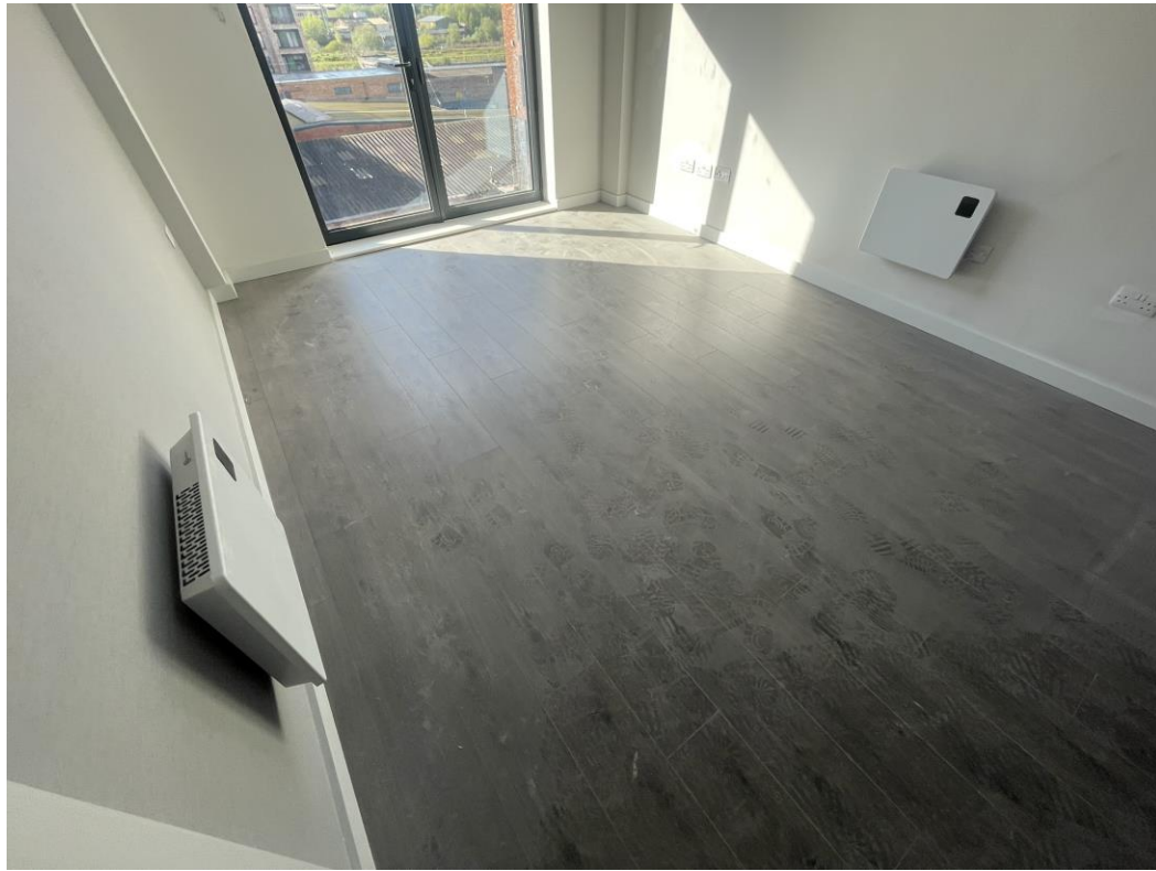
Level 4 – Laminate installed
