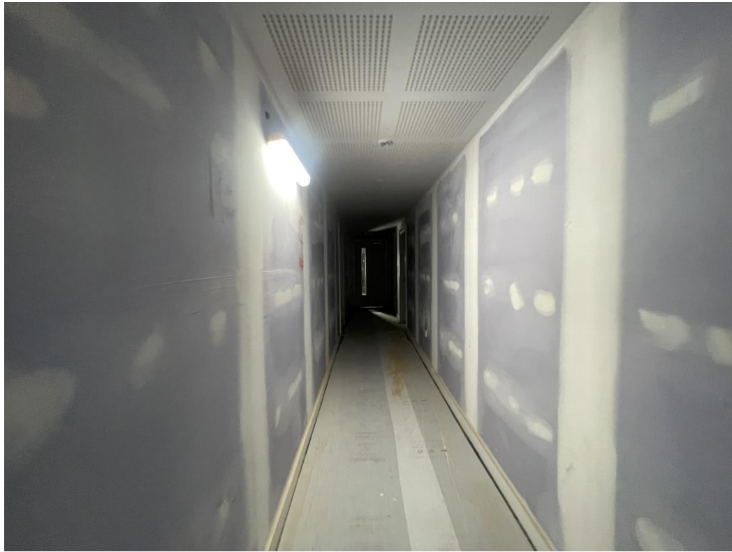
Level 3 – Corridor walls tape & jointed
