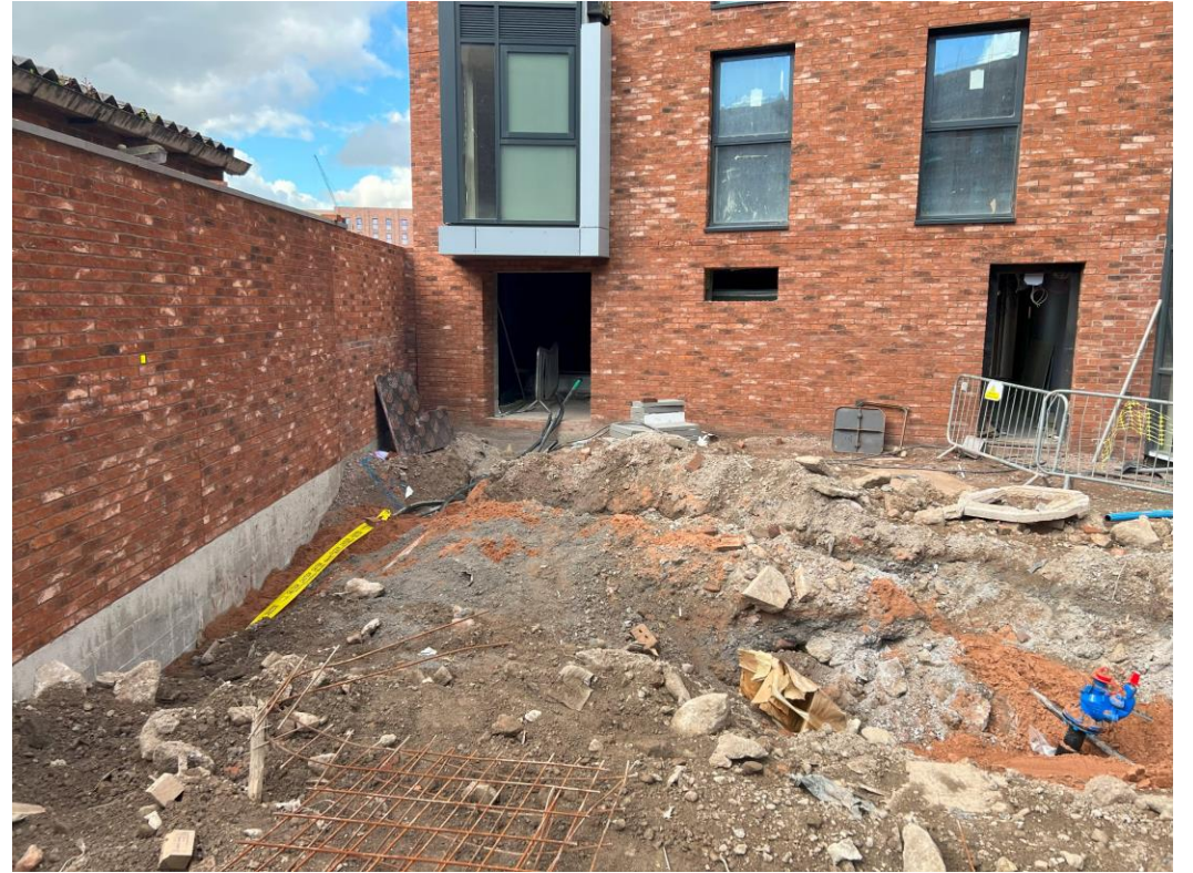
Ground Floor – Mains services installation ongoing
