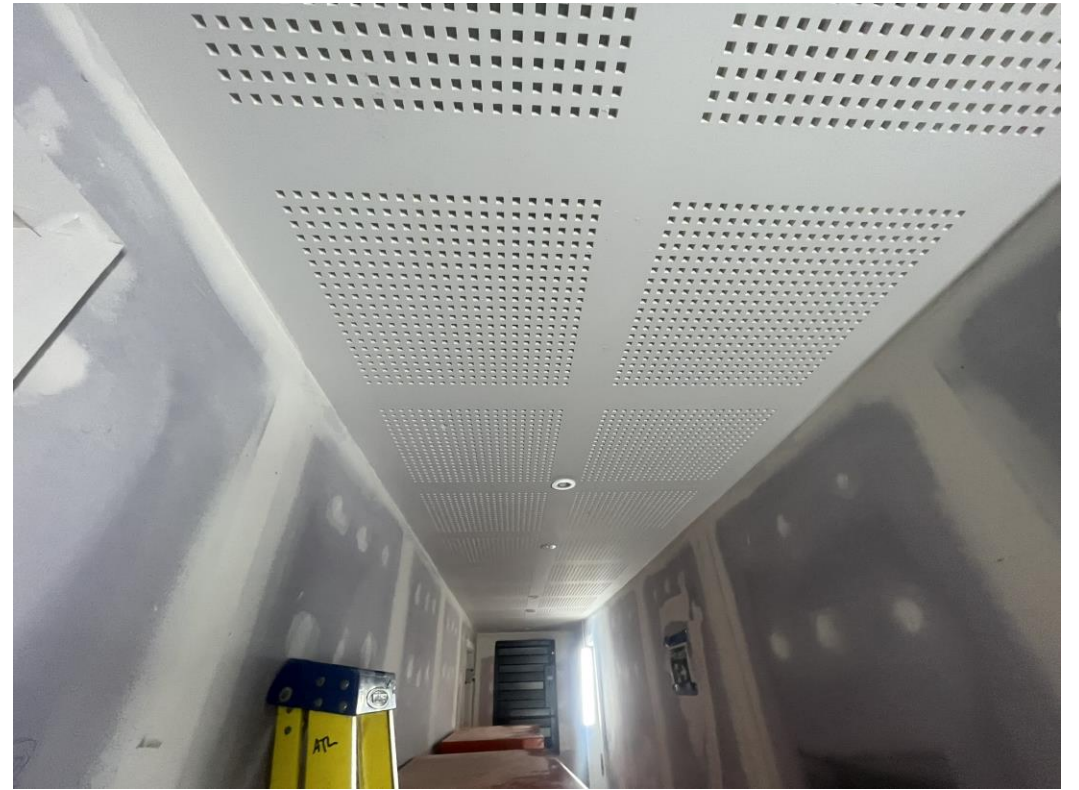
Level 5 – Acoustic ceiling decoration corridor
