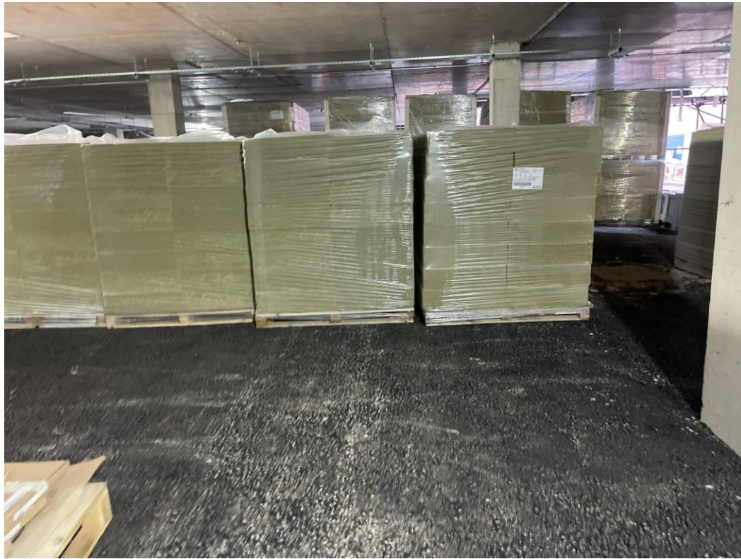
Ground Floor – Soffit insulation loaded for installation
