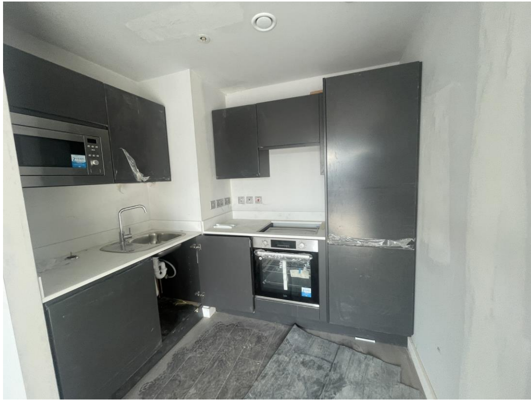
Level 8 – Appliances installed
