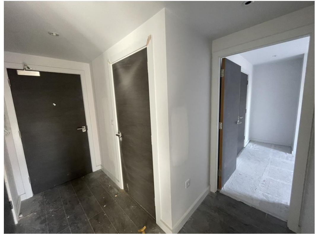
Level 4 – Internal doors installed
