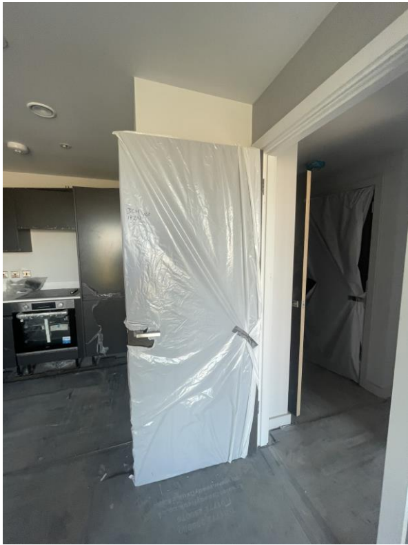
Level 7 – Doors installed
