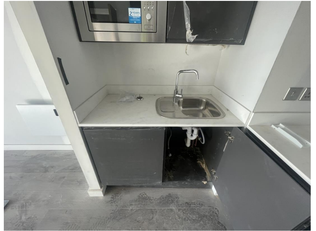
Level 8 – Sink installed
