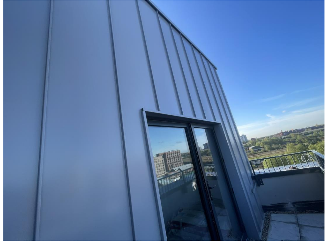
Block A Rainscreen cladding
