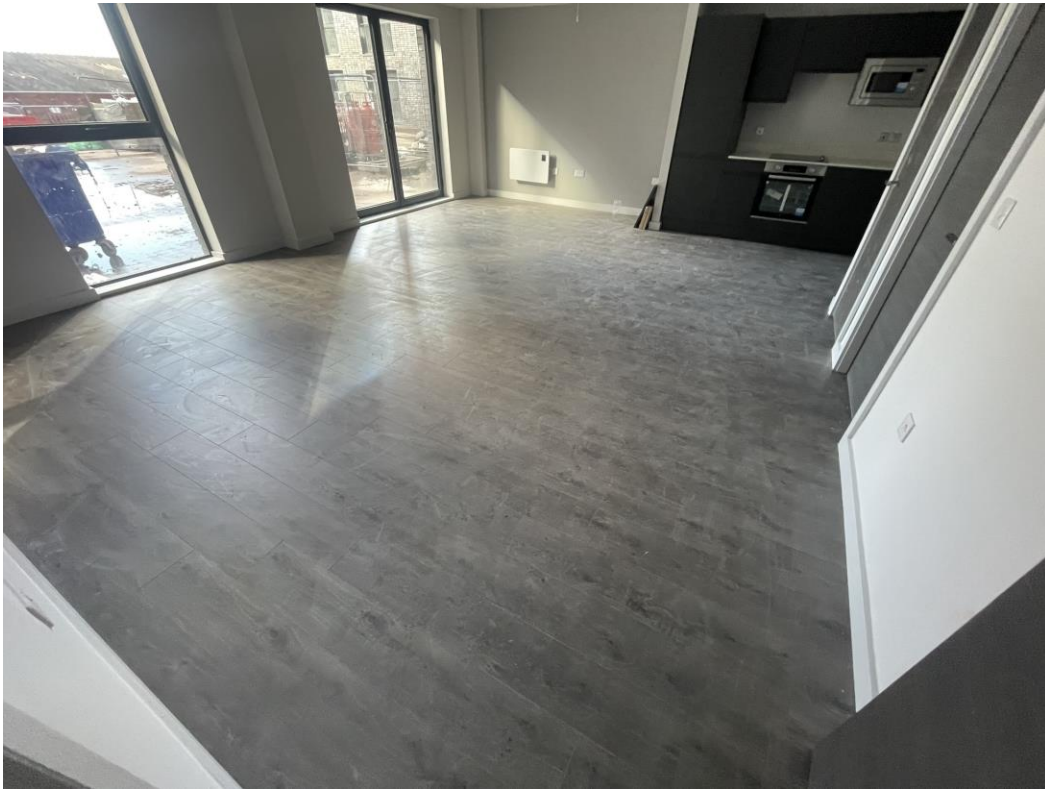
1 st Floor – Laminate installed
