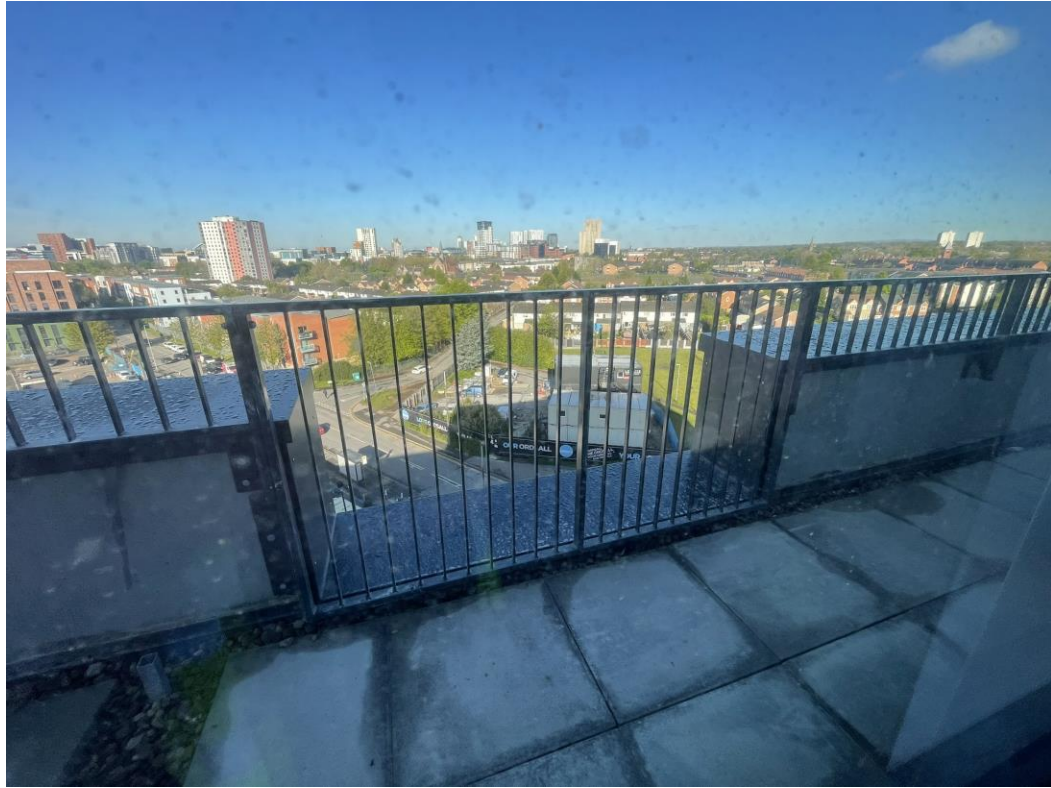
Block A Balustrade handrail
