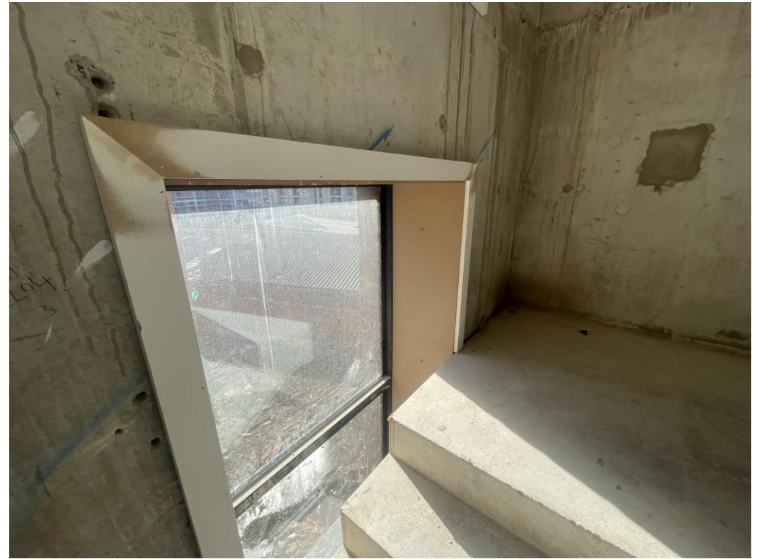
Level 3 – MDF window encasements installation commenced
