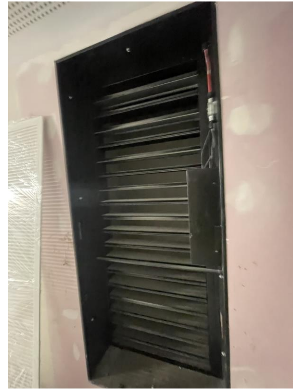
Level 6 – Louvre grills installed
