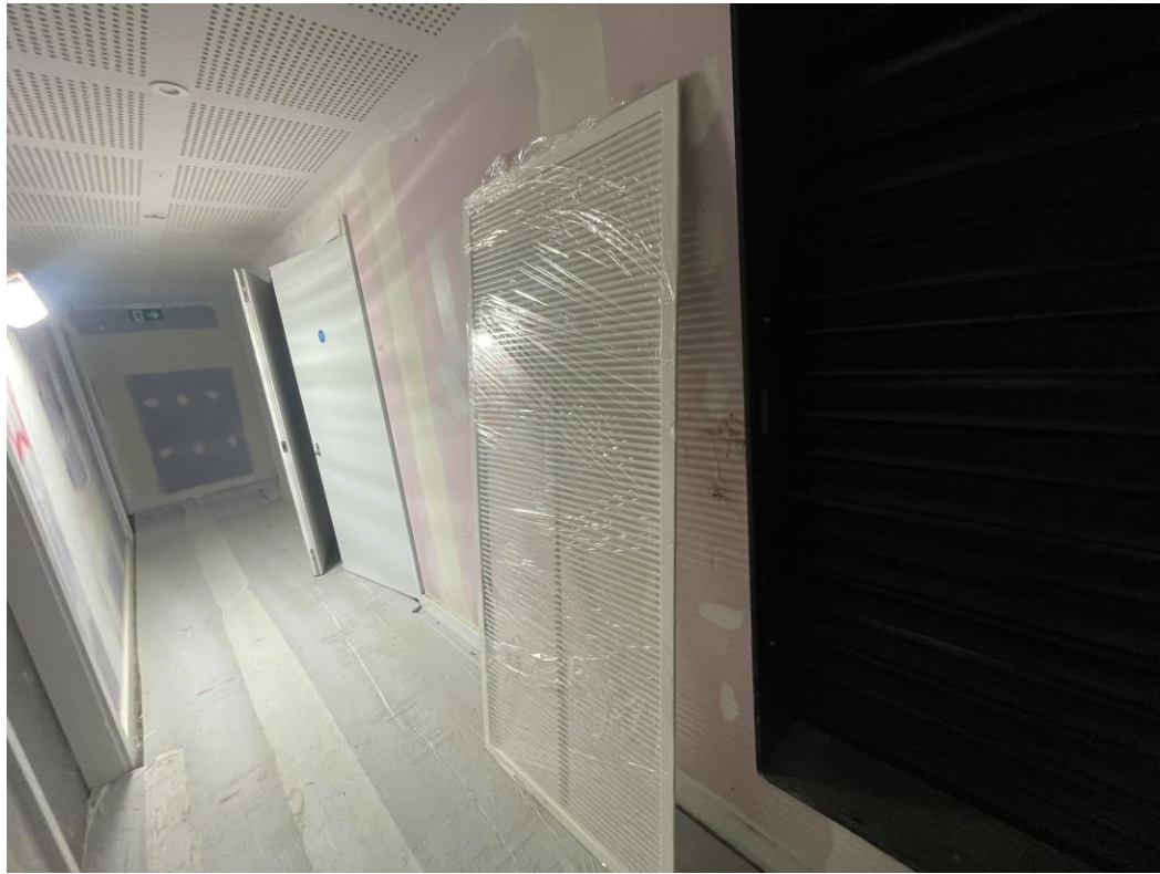
Level 6 – Louvre grills loaded for installation
