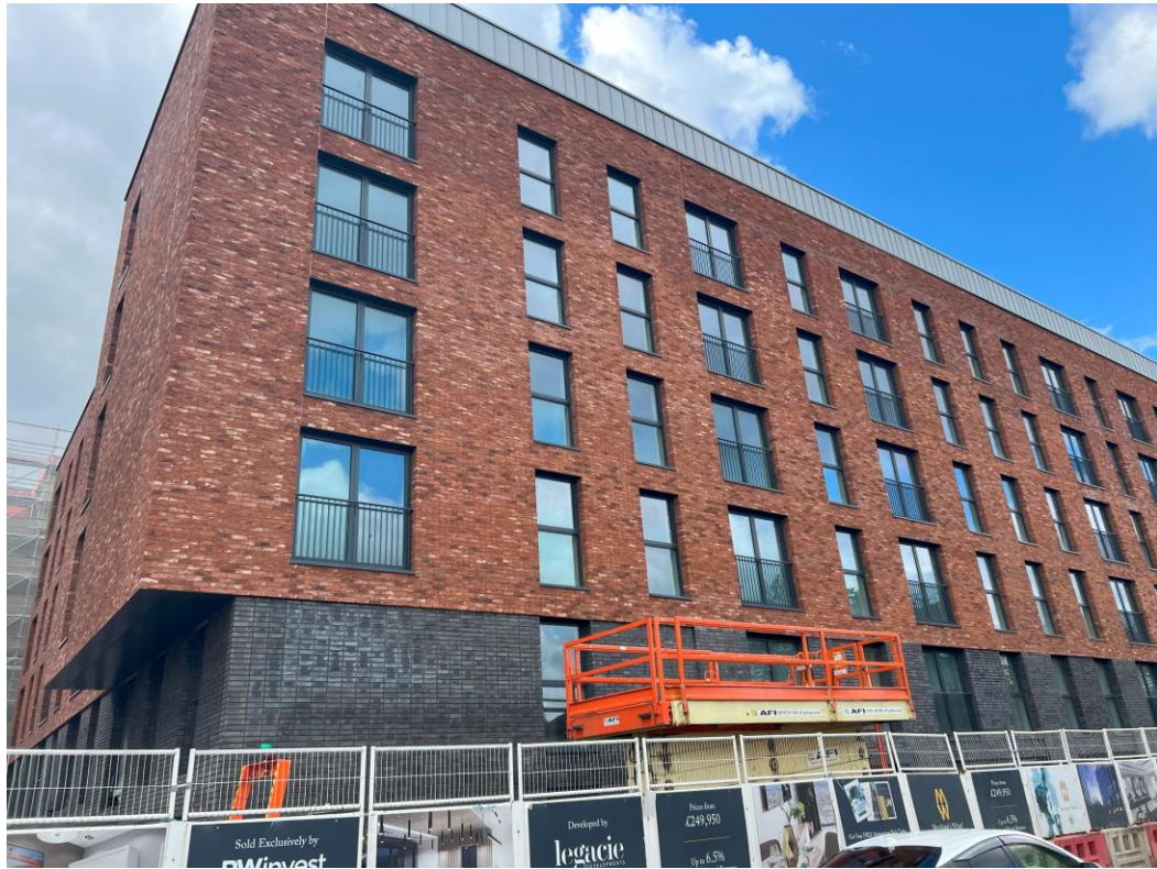
Ordsall Lane site view
