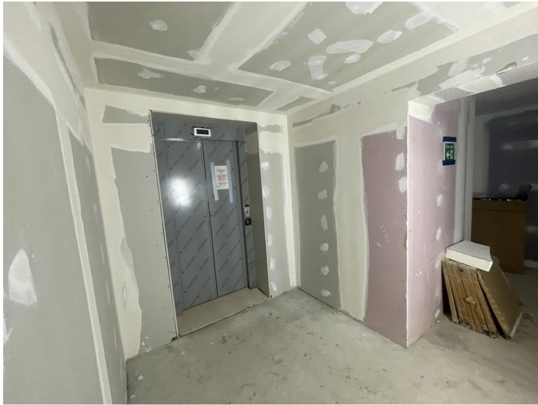
Level 5 – Lift lobby walls & ceiling tape & jointing
