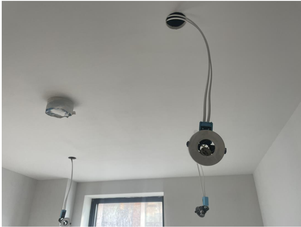
Level 3 – 2 nd fix electrical lighting ongoing
