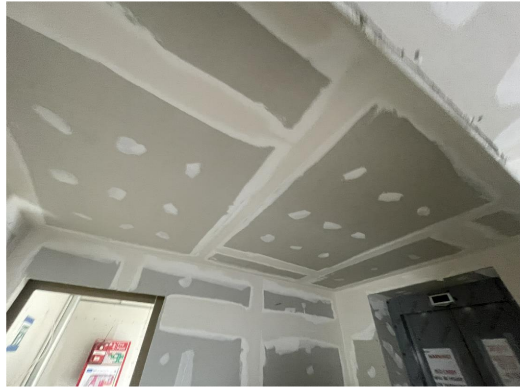
Level 2 – Lift lobby ceiling tape & jointed
