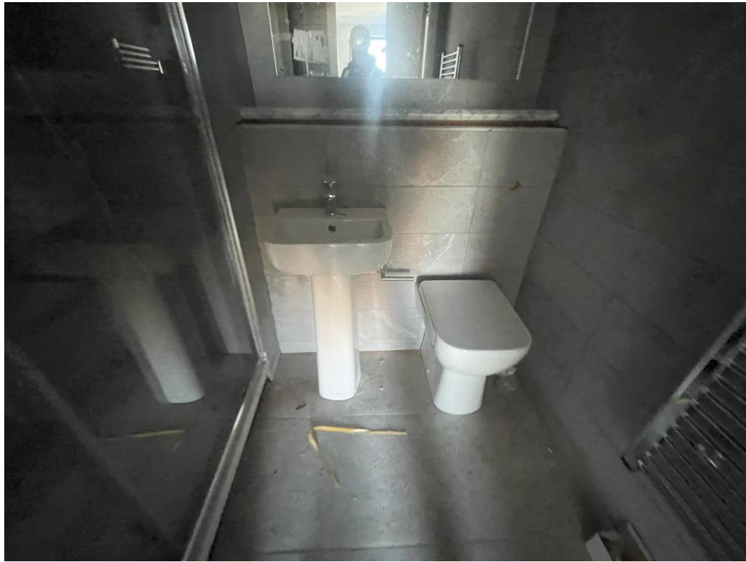
Level 3 – Sanitary items installed
