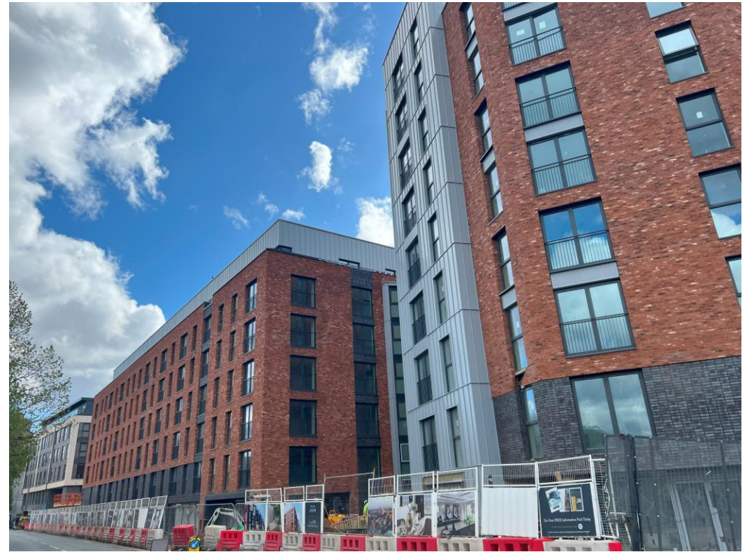
Ordsall Lane site view
