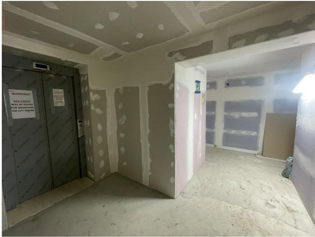
Level 2 – Lift lobby walls tap & jointed
