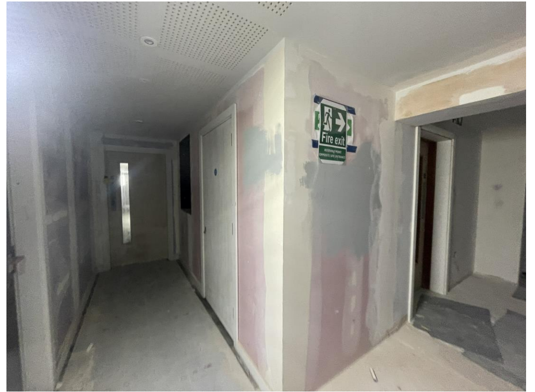
Level 3 – Corridor walls tape & jointed
