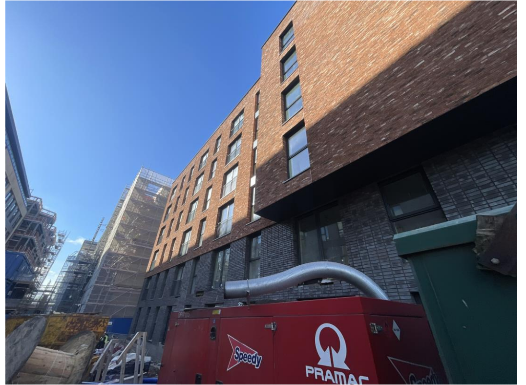
Ordsall Lane site view
