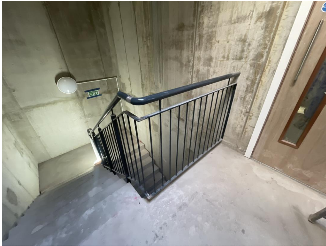
Level 6 - Stairwell balustrades
