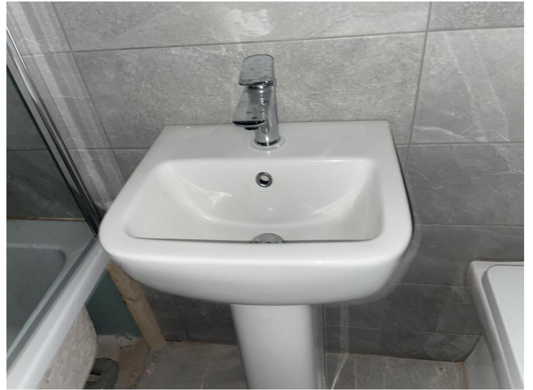
Level 5 - Bathroom sanitary items installed
