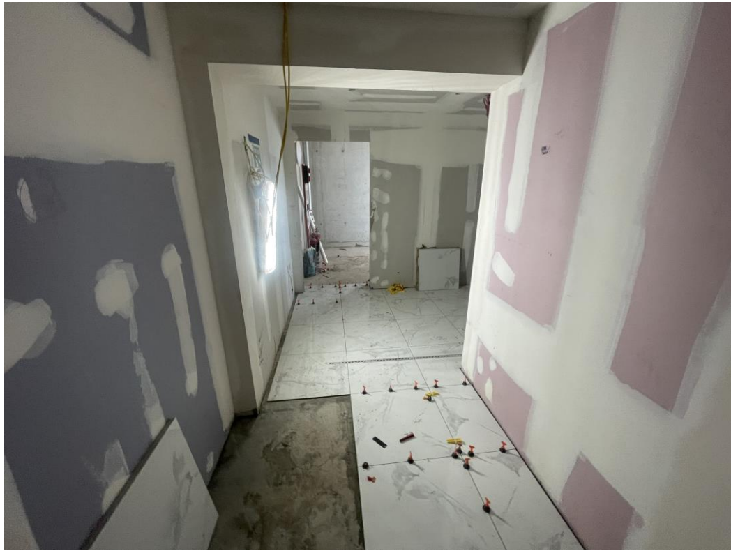
Level 6 – Floor tiling ongoing
