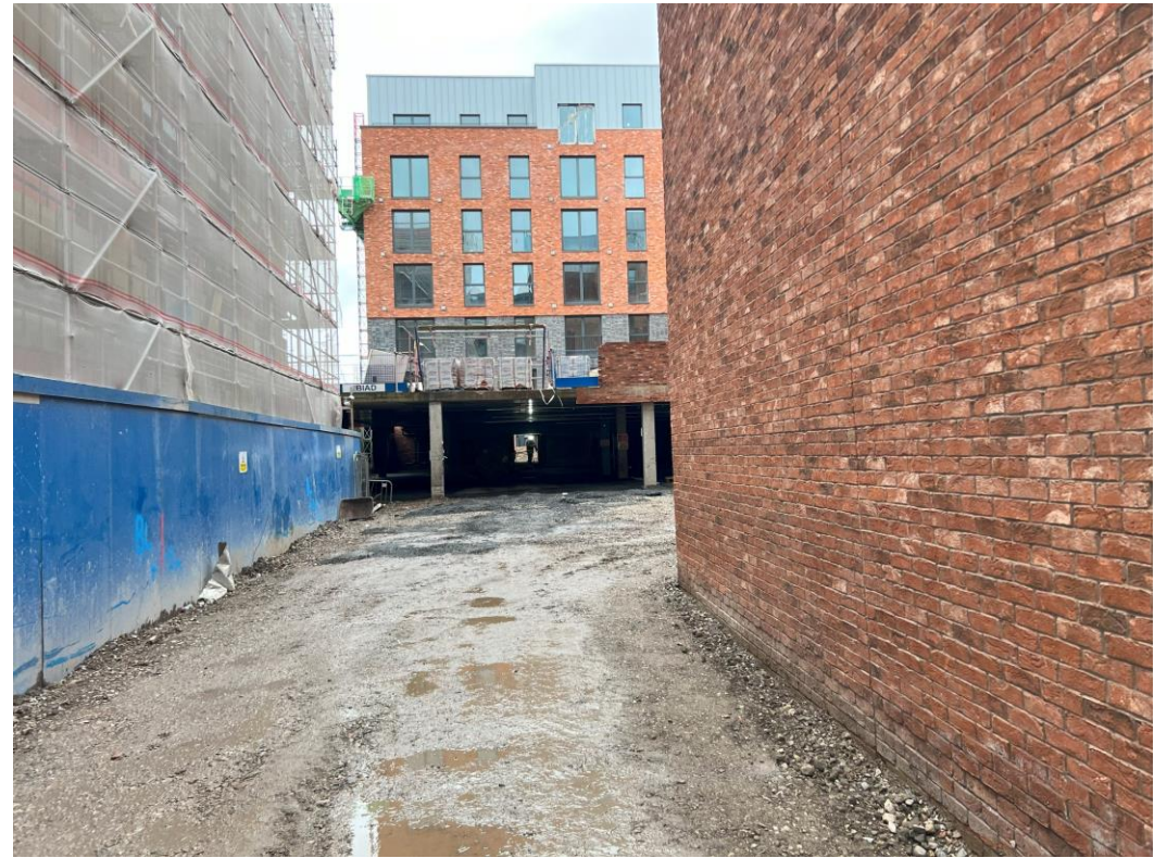
Podium site view
