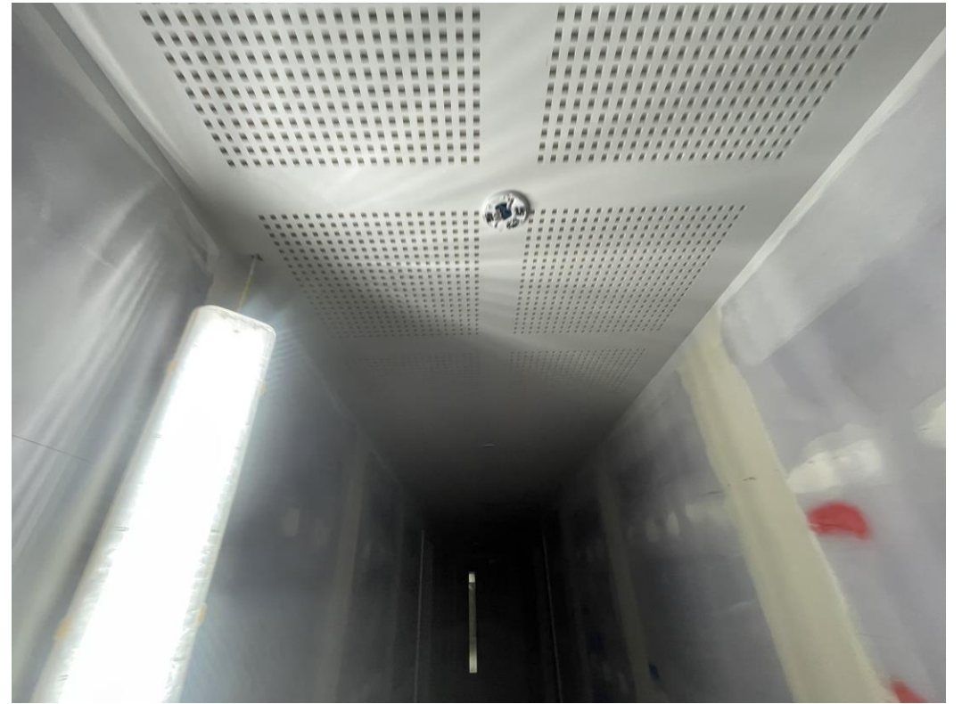
Level 6 – Acoustic ceiling decoration corridor
