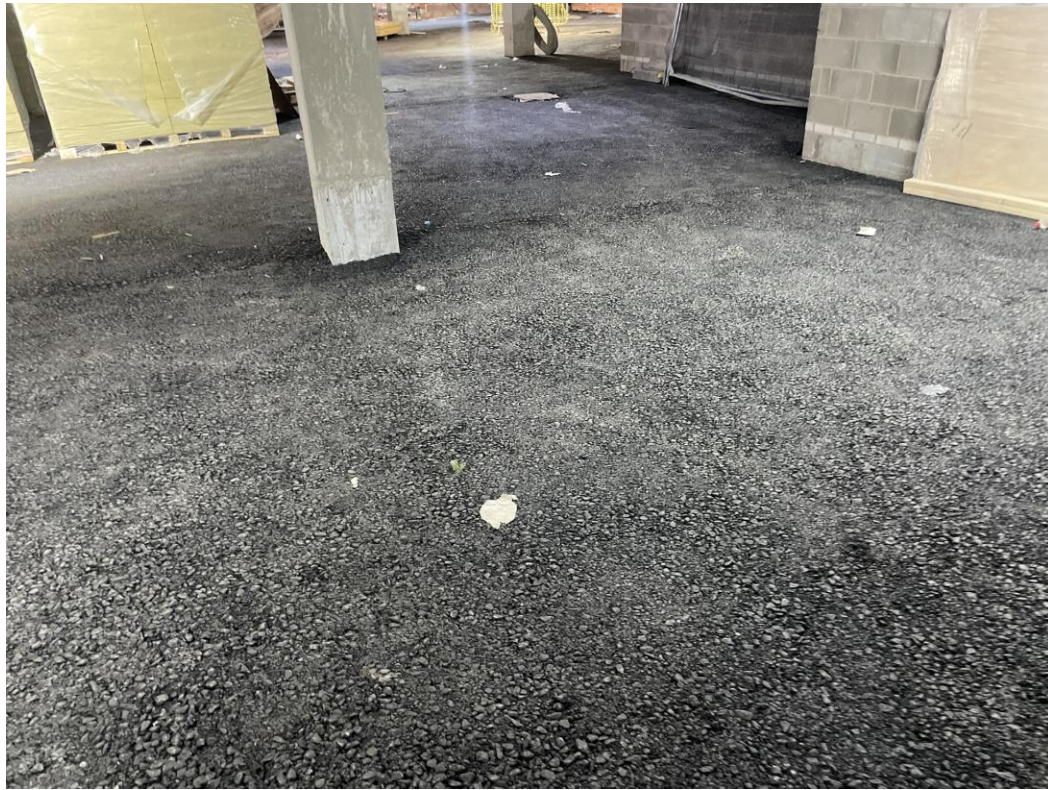
Ground Floor - Ground works ongoing
