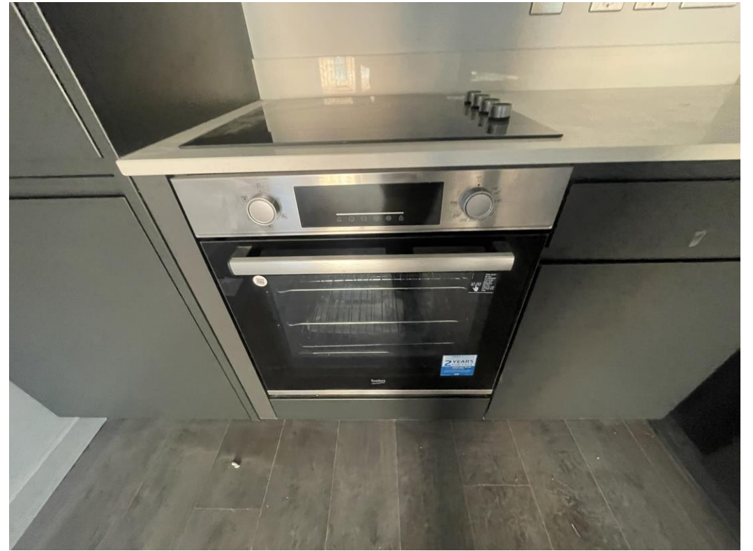
Level 2 – kitchen appliances installed
