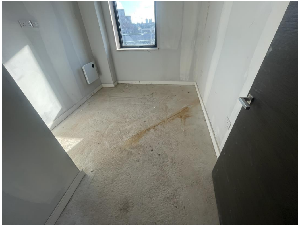
Level 8 – 2 nd fix joinery
