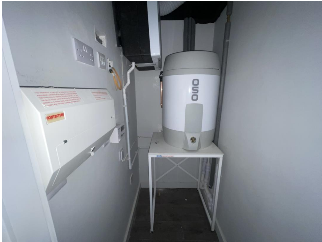
Level 3 – 2 nd fix mechanical & electrical
