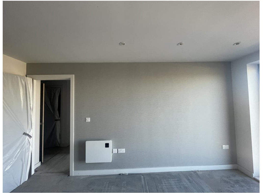
Level 7 – Feature wall installed
