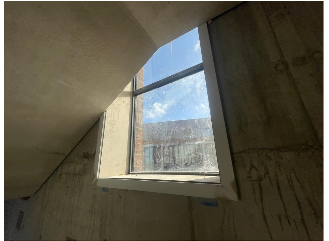
Level 4 – MDF window encasements installation commenced
