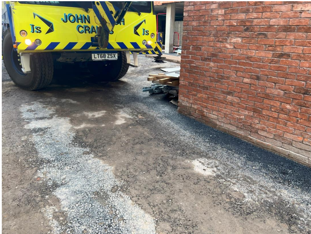
Tarmac works ongoing
