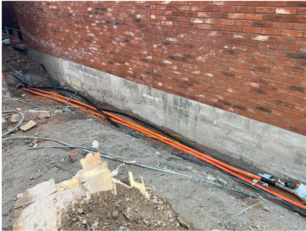
Ground Floor – Mains services installation ongoing
