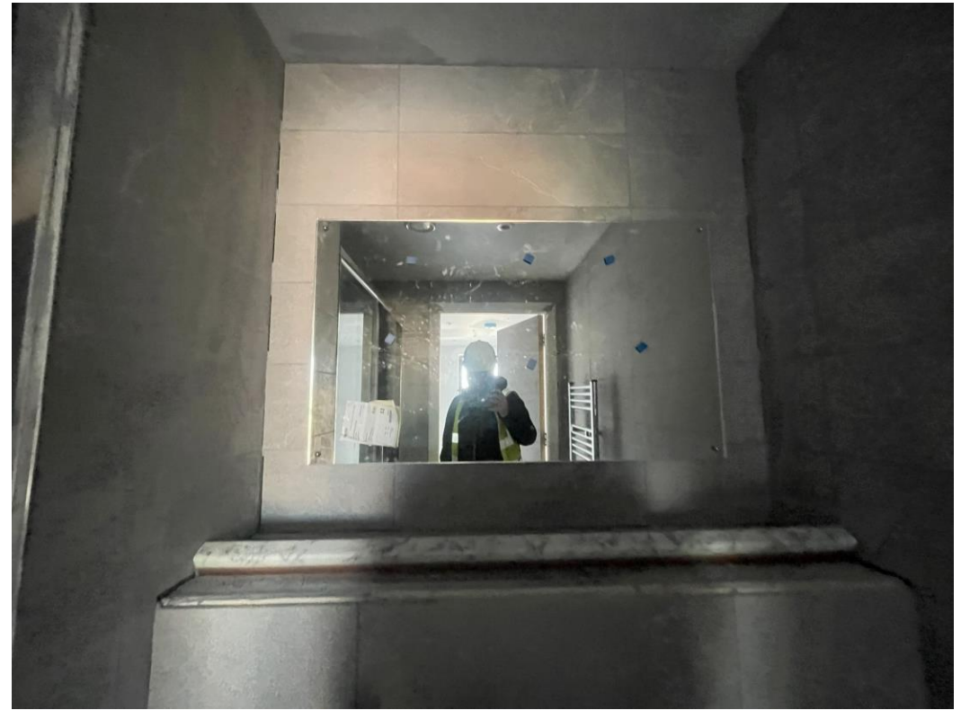
Level 3 – Bathroom mirror installed
