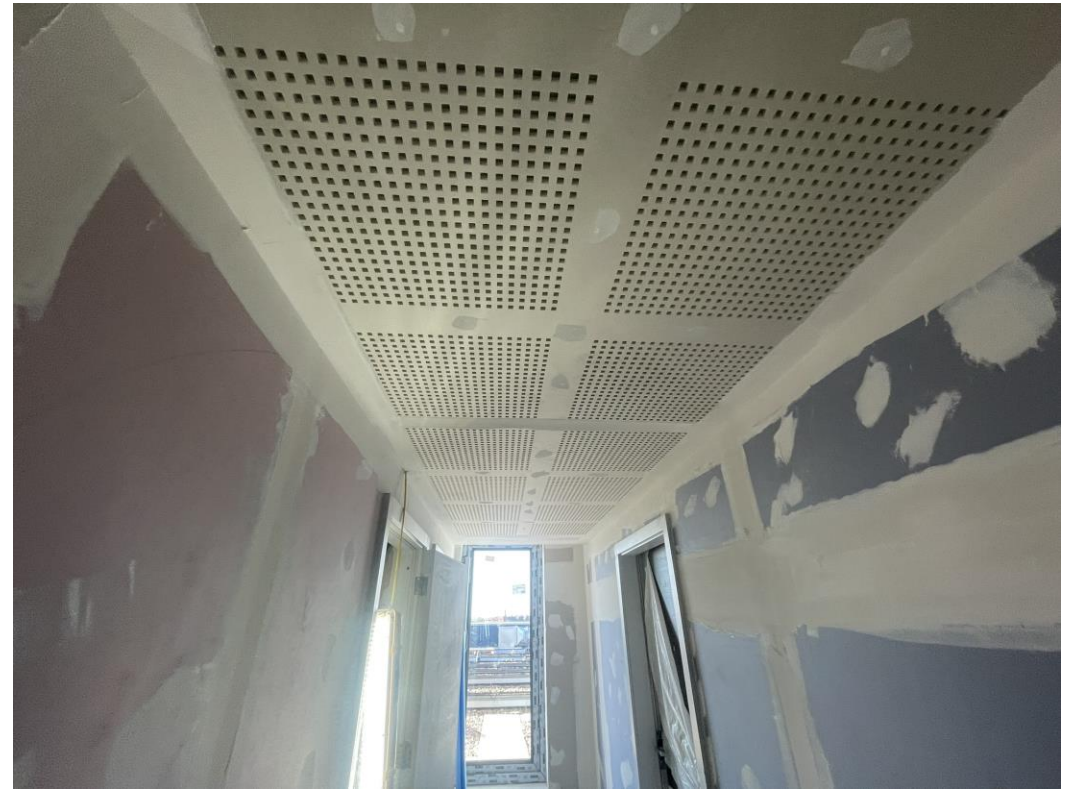
Level 7 – Acoustic ceiling decoration corridor
