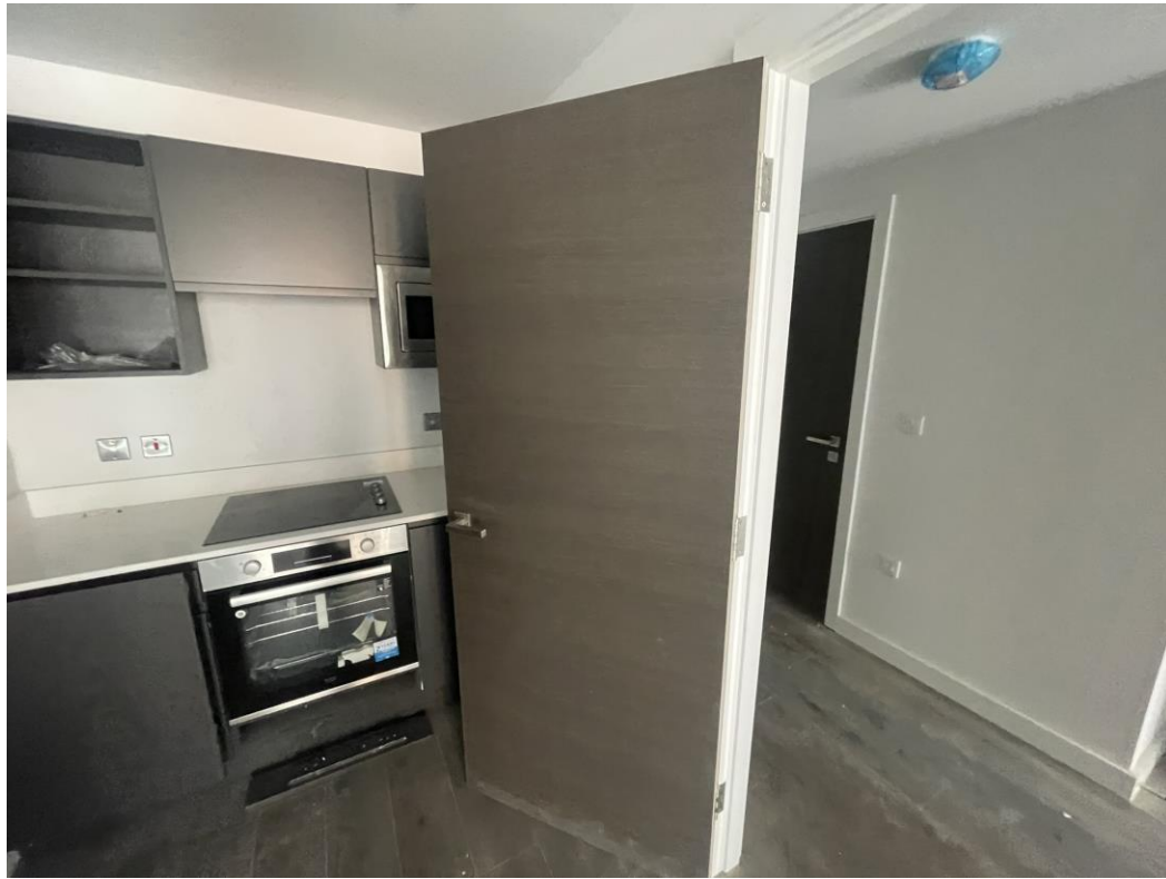
Level 5 – Internal doors installed
