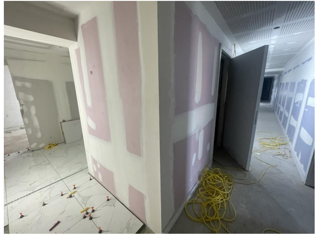
Level 6 – Wall tap & jointing
