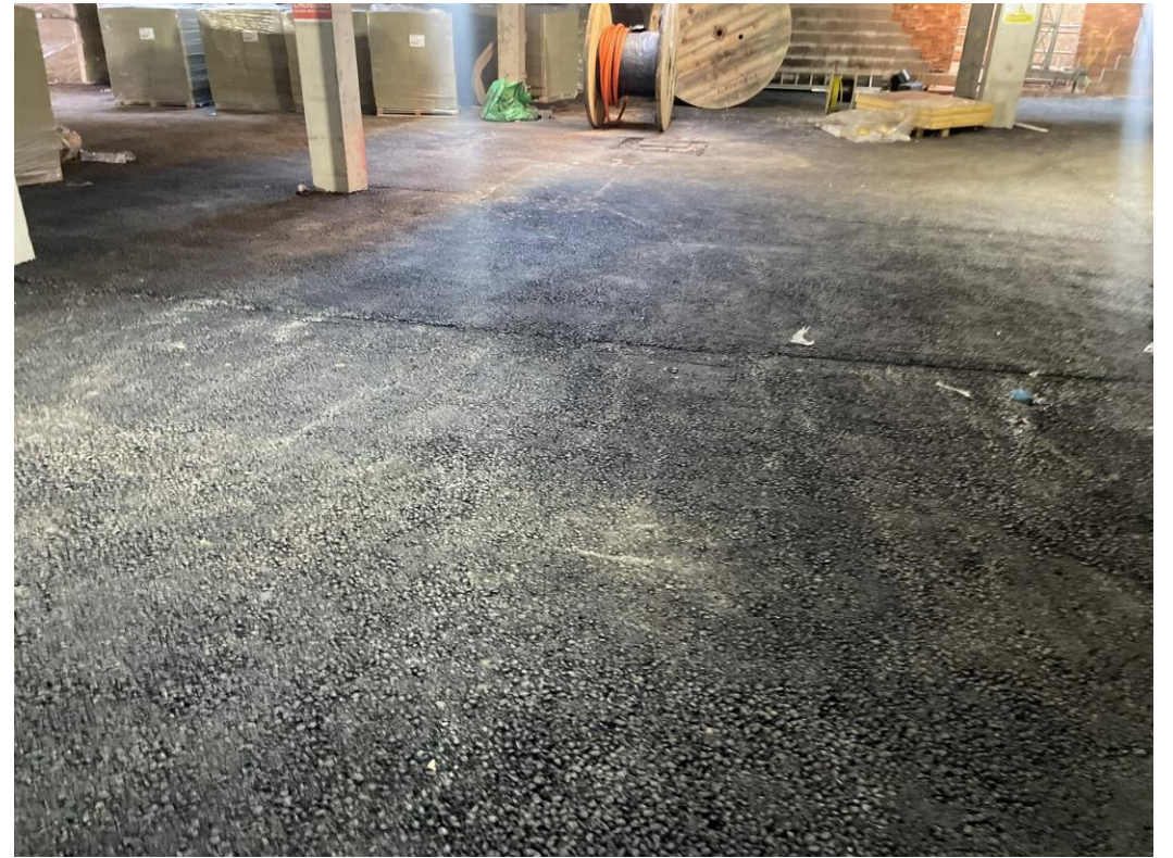
Ground Floor - Ground works ongoing
