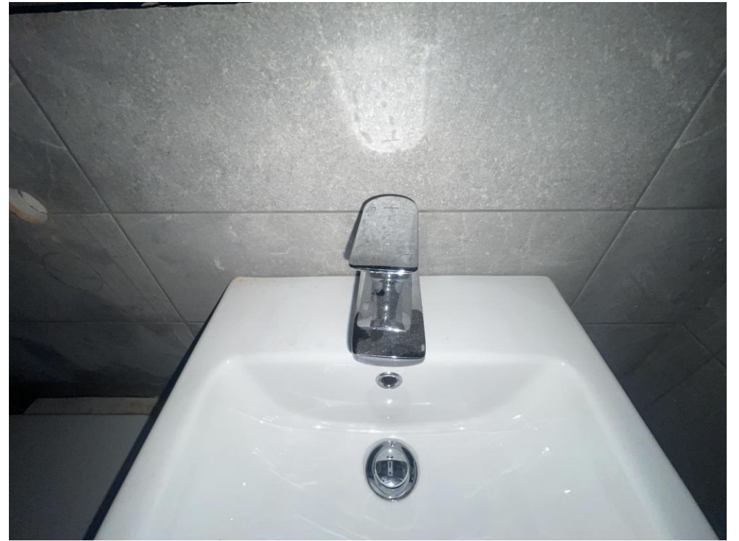
Level 6 – Sanitary items installed
