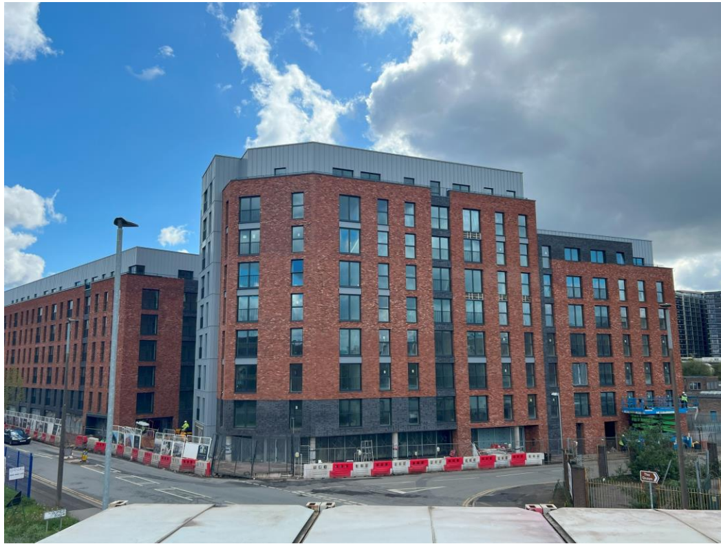
Ordsall Lane site view
