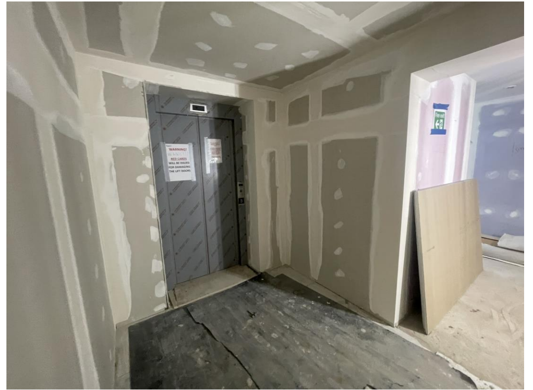
Level 3 – Lift lobby wall & ceilings tape & jointed
