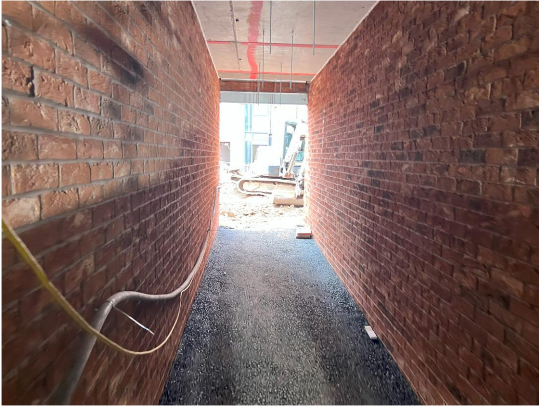
Ground Floor – Tarmac paving to undercroft
