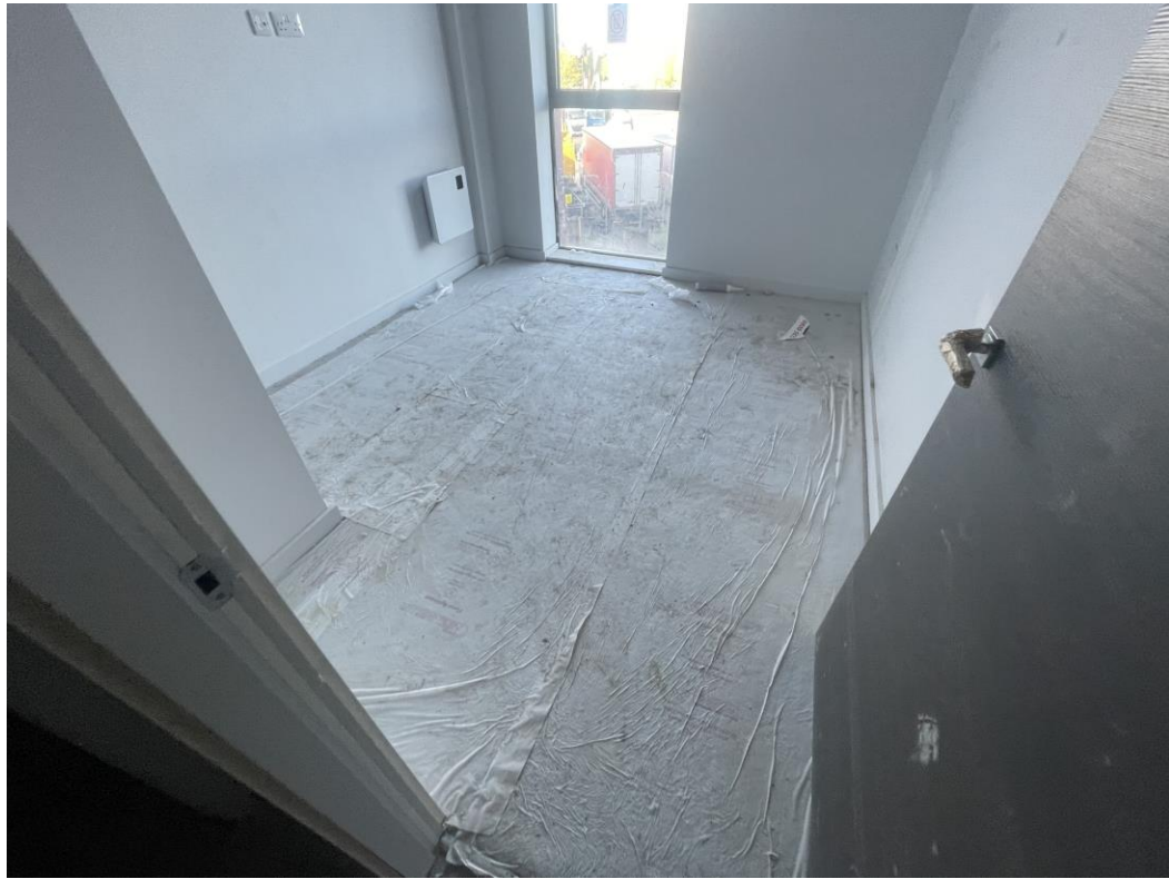
Level 2 – bedroom carpets installed
