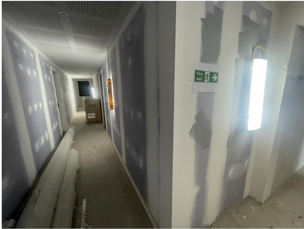
Level 3 – Corridor walls tape & jointed
