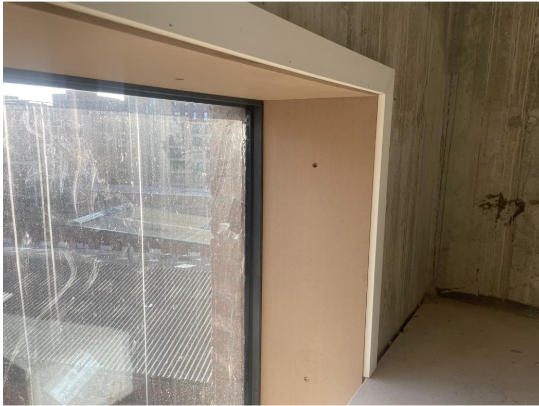
Level 5 – MDF window encasements installation commenced
