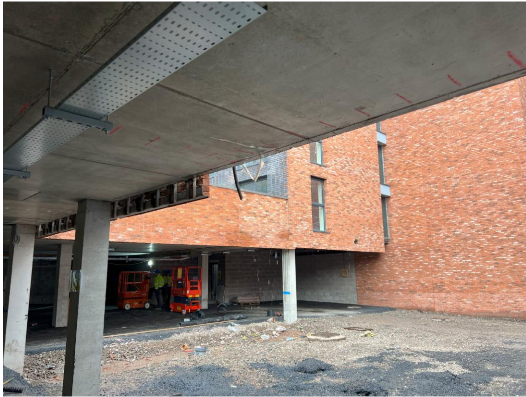
Podium site view
