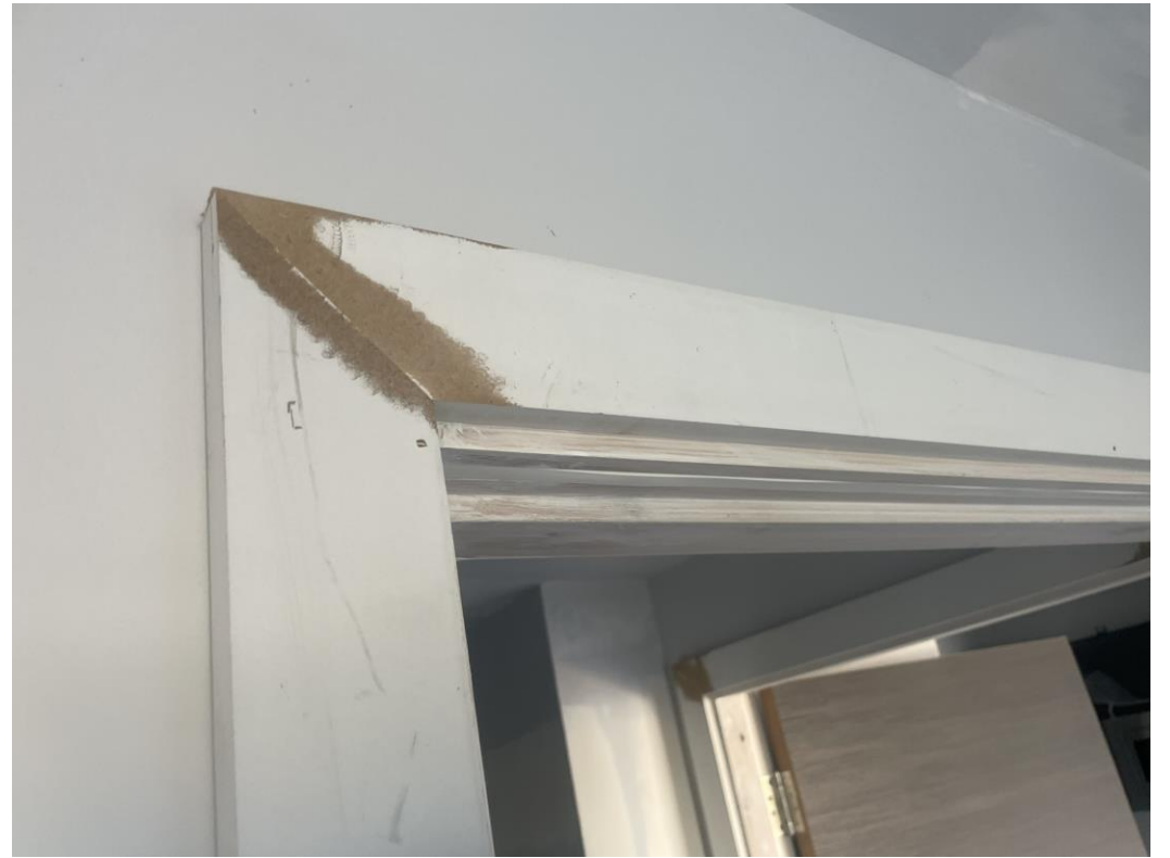
Level 3 – 2 nd fix joinery decoration ongoing
