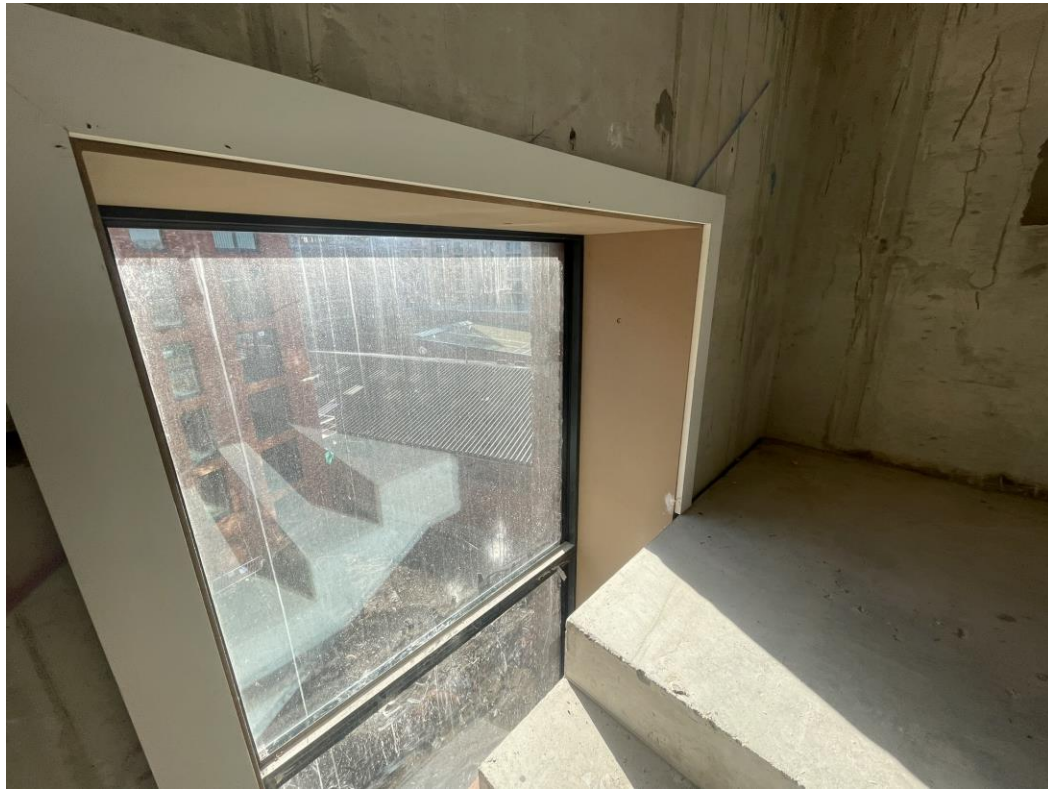
Level 4 – MDF window encasements installation commenced
