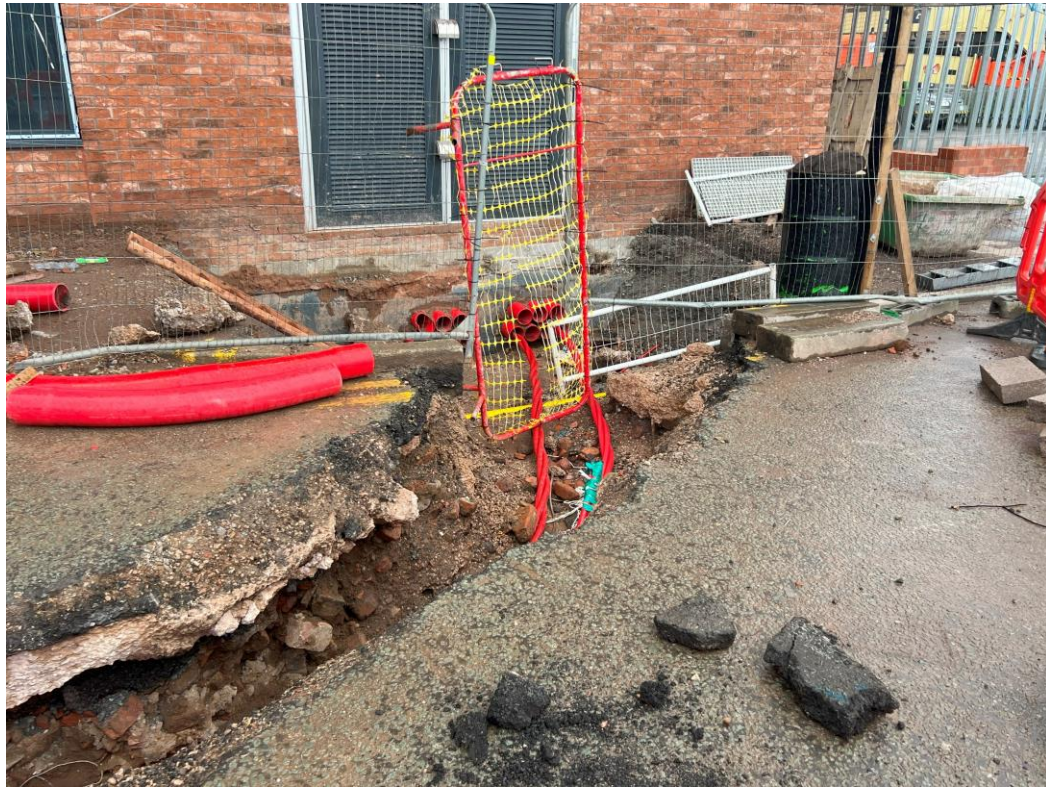
Ground works ongoing
