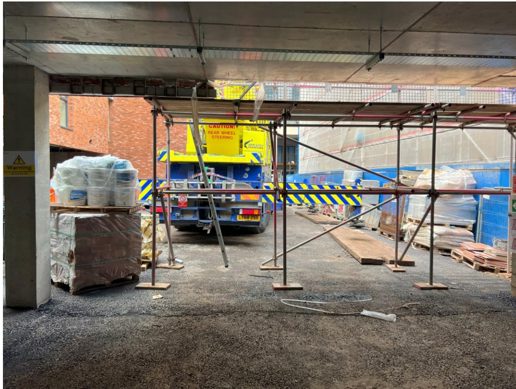
Ground Floor – Tarmac paving to undercroft
