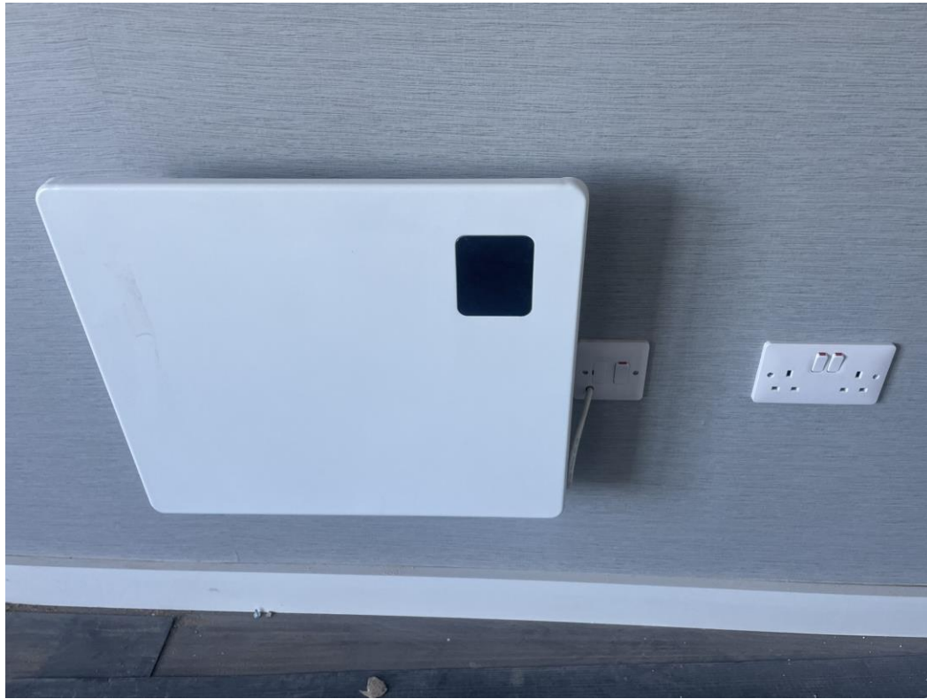
Level 6 – Wall heating panel installed
