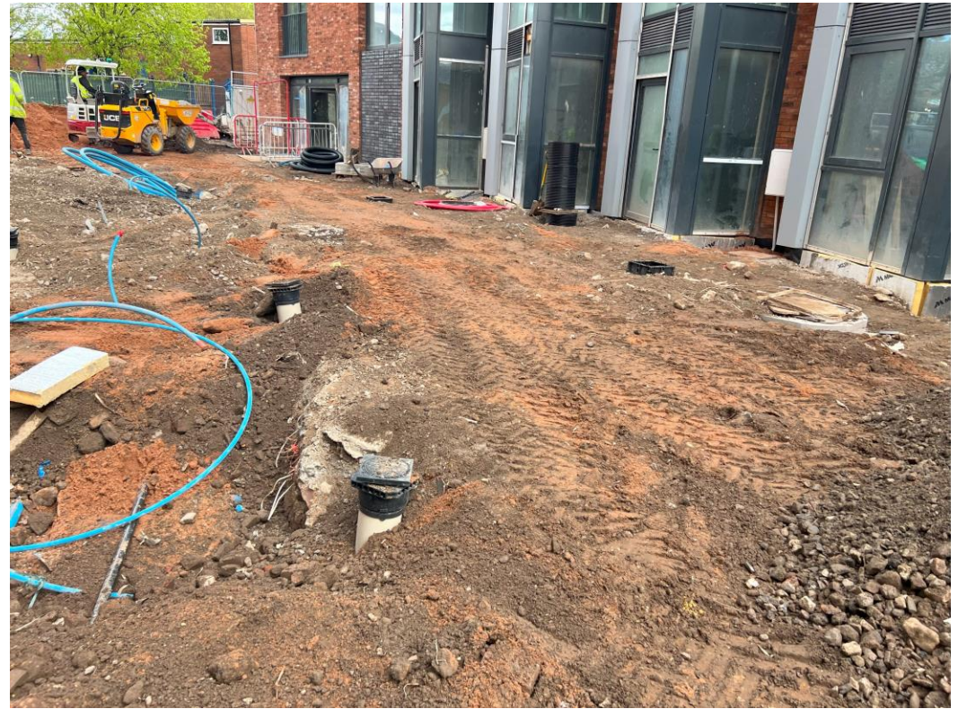
Ground Floor – Mains services installation ongoing
