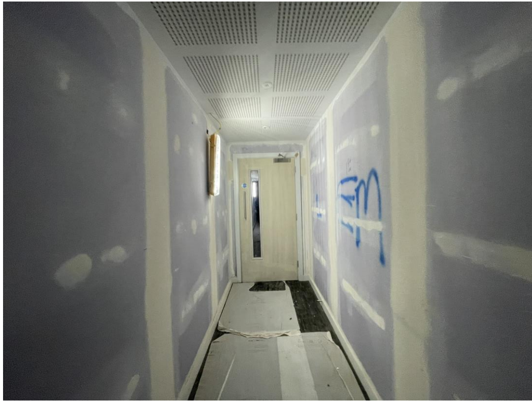
Level 6 – Circulation doors installed
