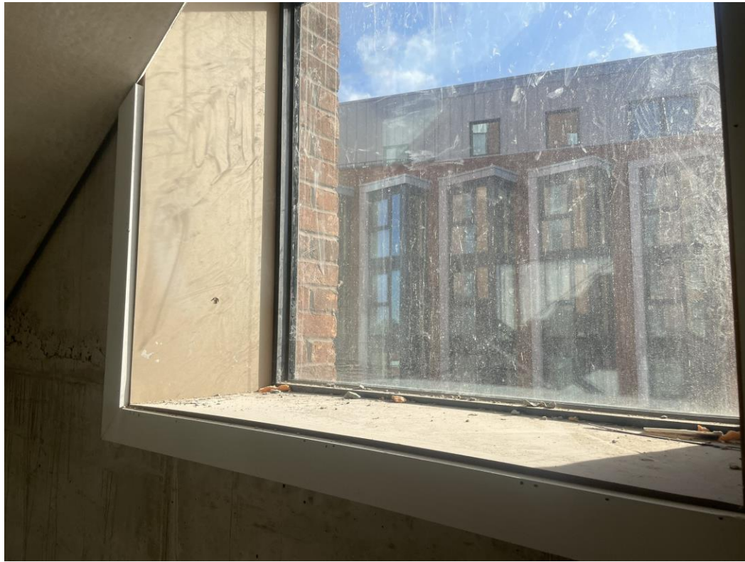
Level 3 – MDF window encasements installation commenced
