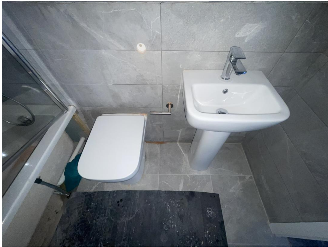
Level 6 – Sanitary items installed
