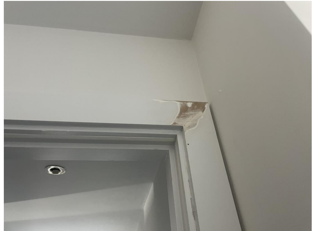
Level 5 – 2 nd Fix joinery decoration ongoing
