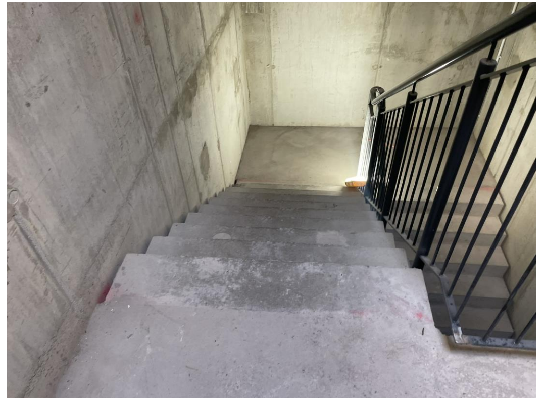
Level 6 - Stairwell balustrades
