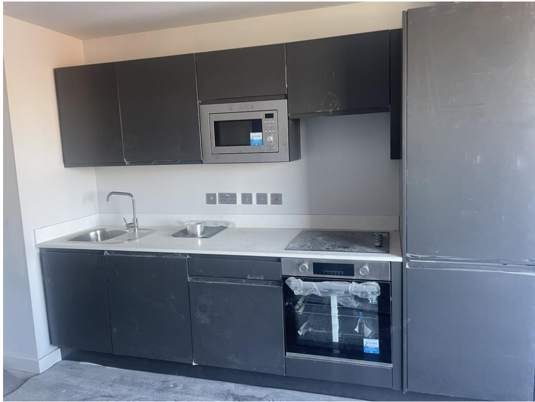
Level 6 – Kitchen complete
