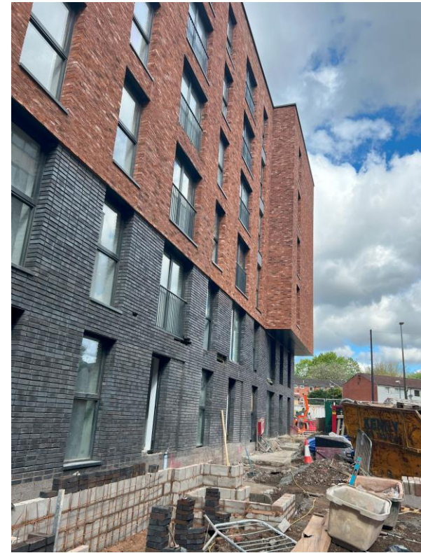
Ordsall Lane site view
