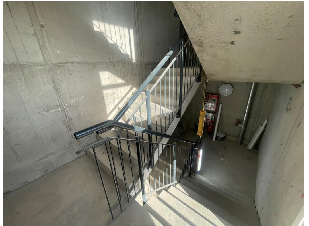
Block A – Balustrades installed
