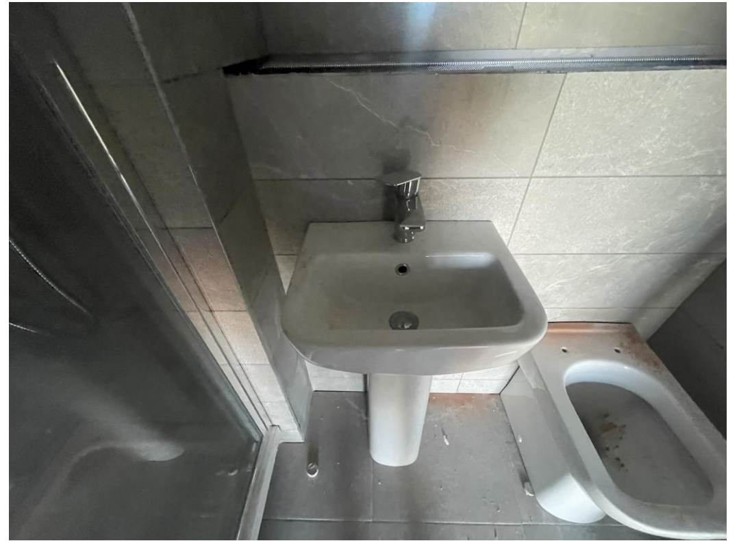
Level 5 – Sanitary items installed
