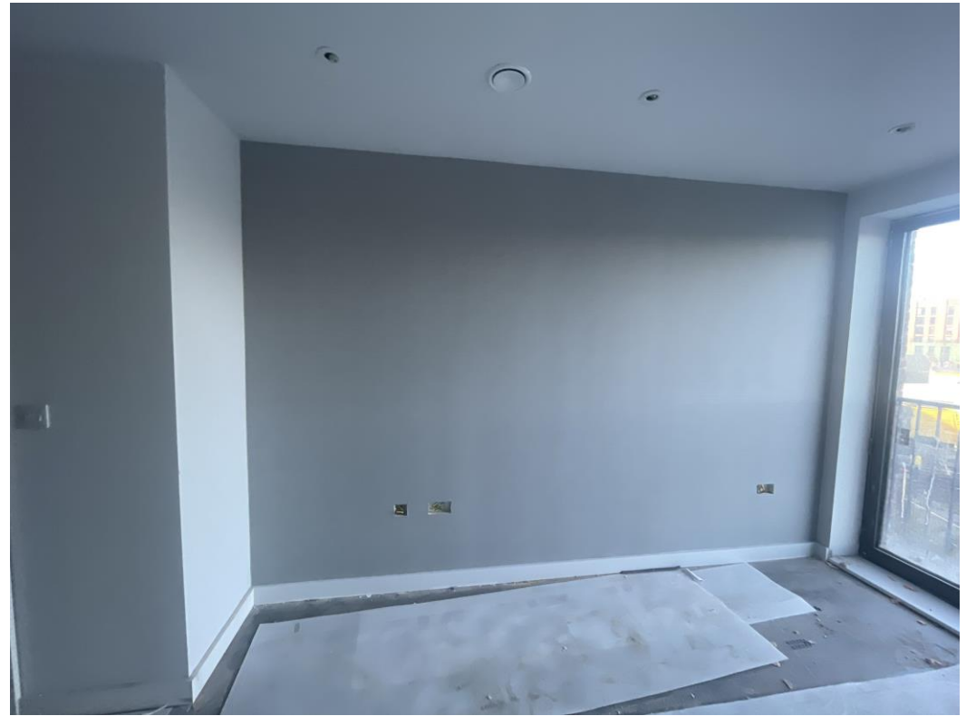
Level 2 – Feature wall installed
