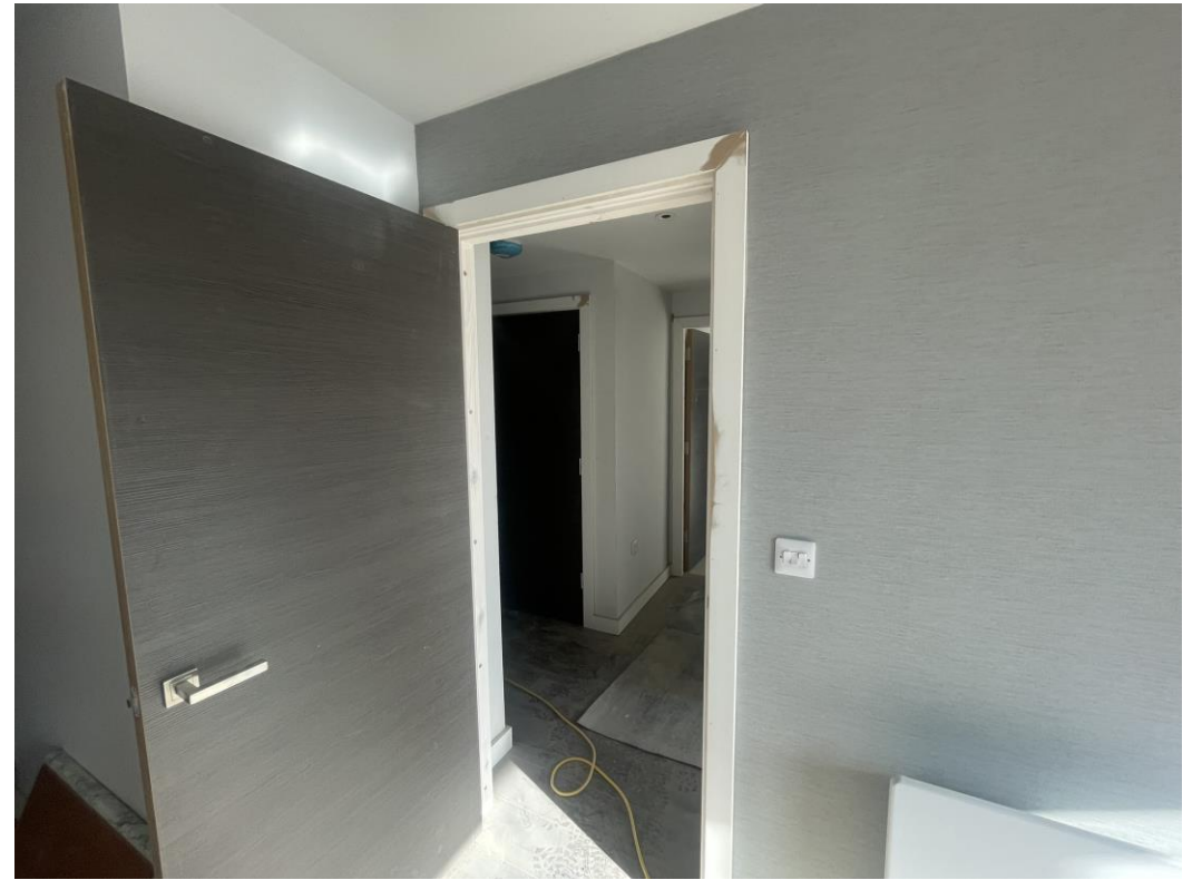
Level 6 – 2 nd Fix joinery decoration ongoing
