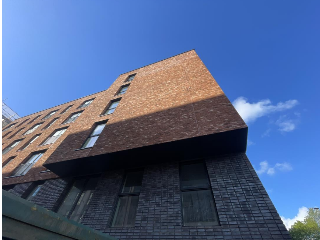
Ordsall Lane site view
