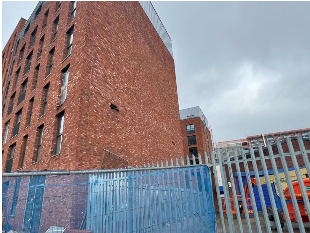
Block A – Viewed from Worrall Street
