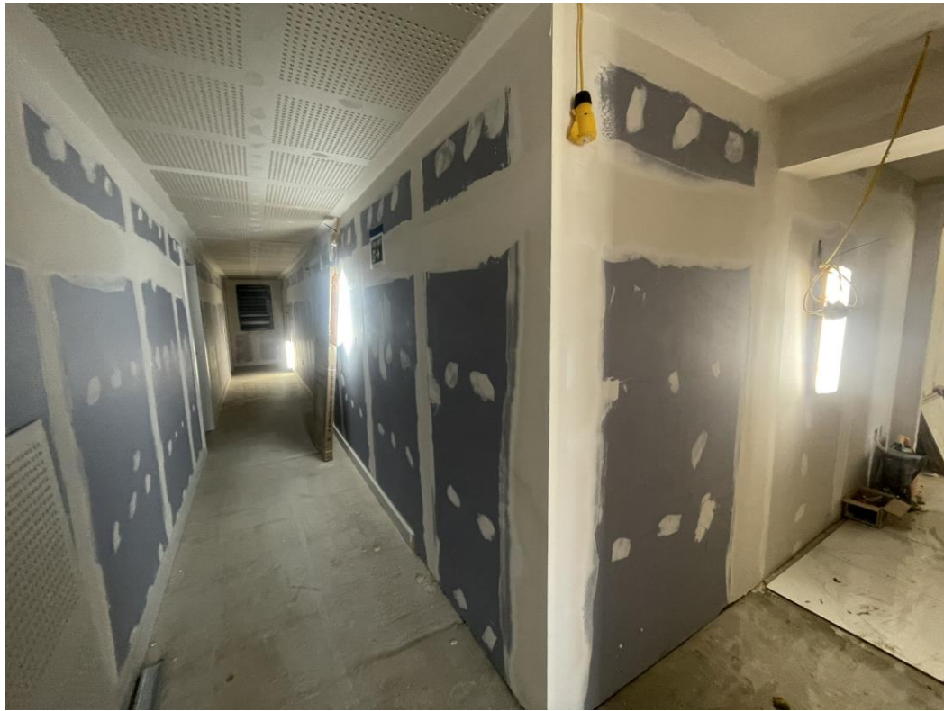
Level 7 – Tape & jointing to walls ongoing
