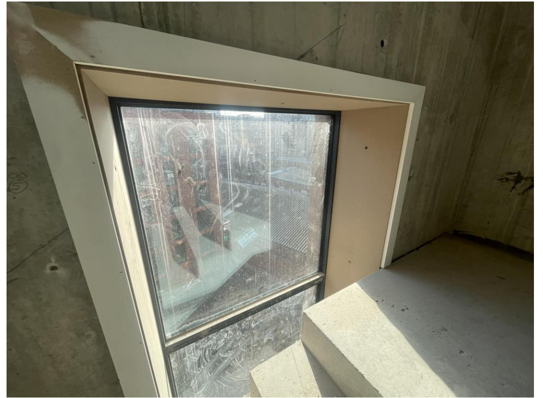
Level 5 – MDF window encasements installation commenced
