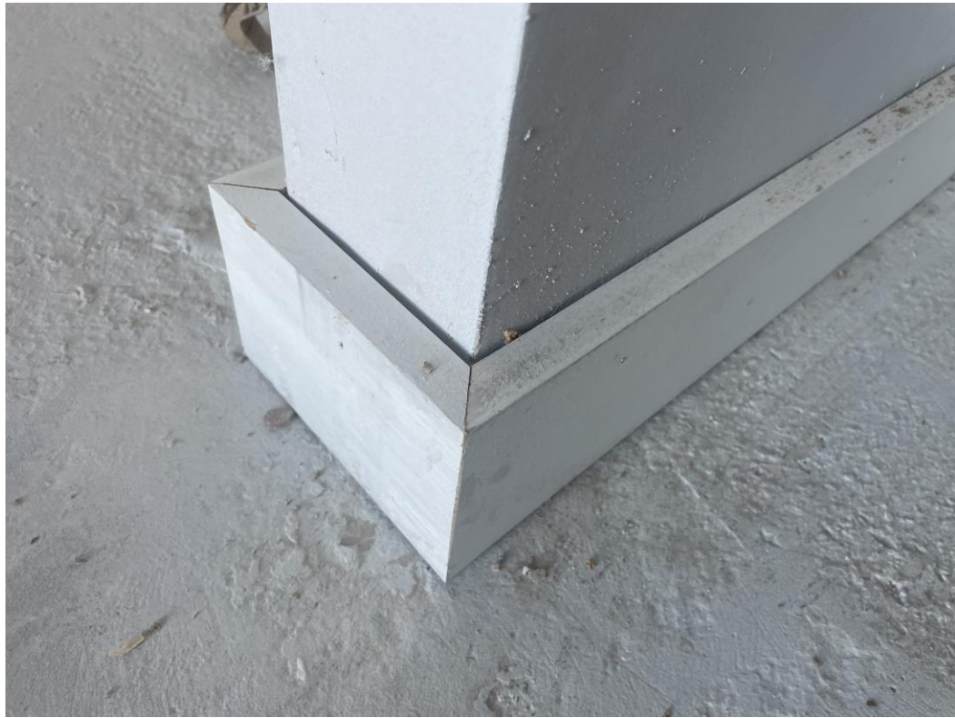
Level 3 – 2 nd Fix joinery installed
