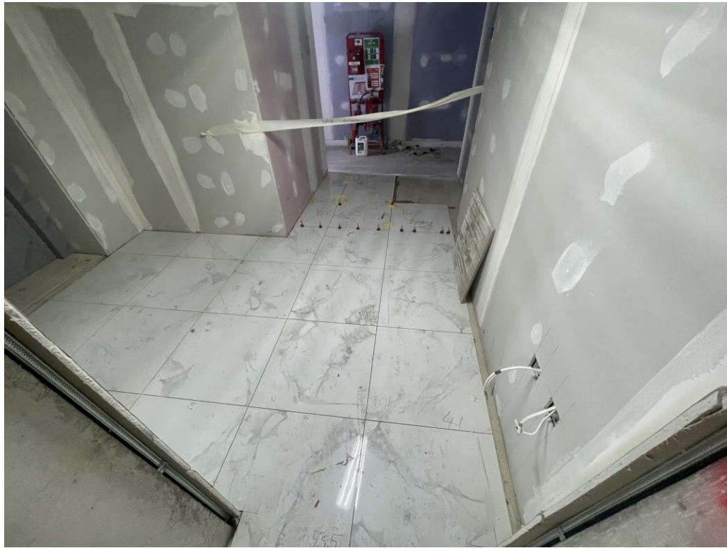
Level 4 – Lift lobby floor tiling
