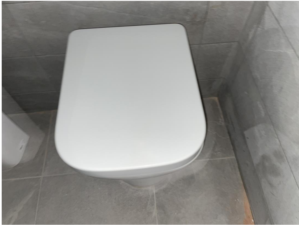
Level 5 - Bathroom sanitary items installed
