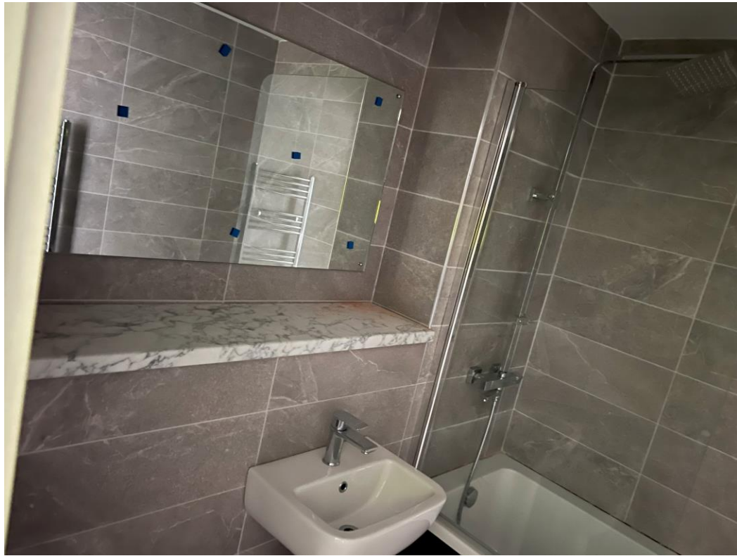
Level 4 – Bathroom mirror installed
