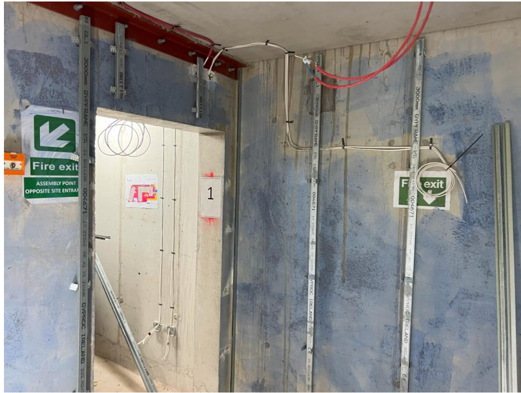
Block A – Partition work to staircase has commenced
