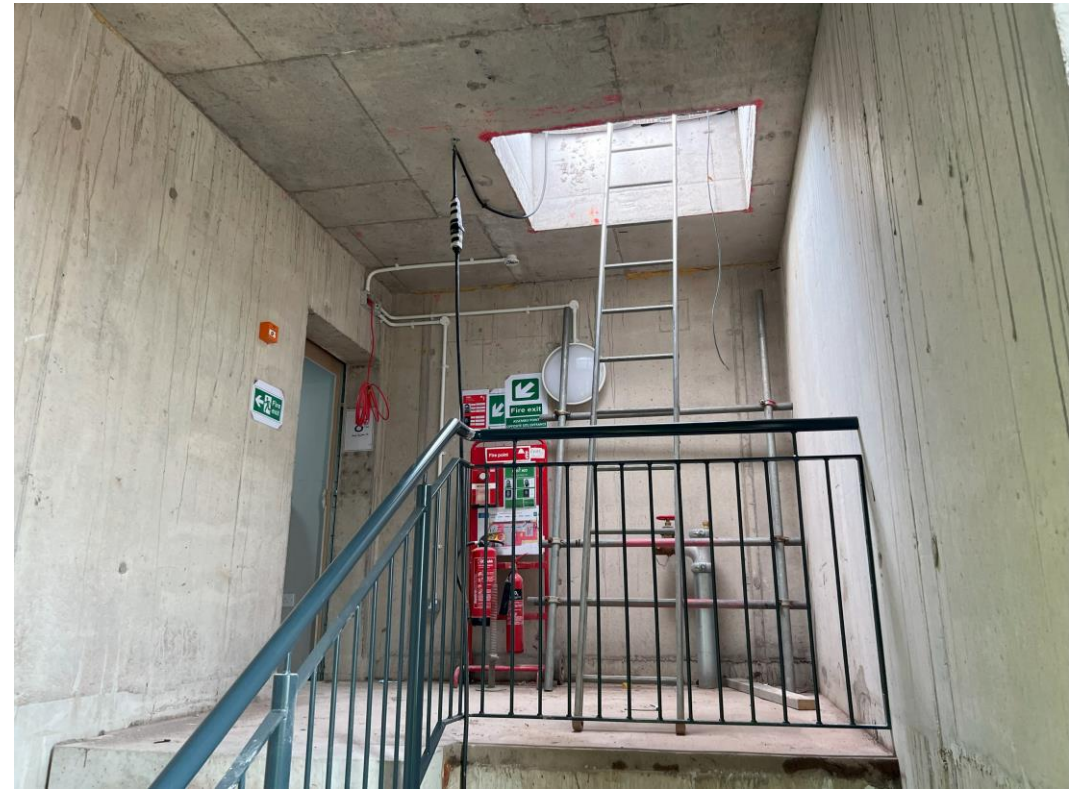
Block A – Handrail & balustrade installed
