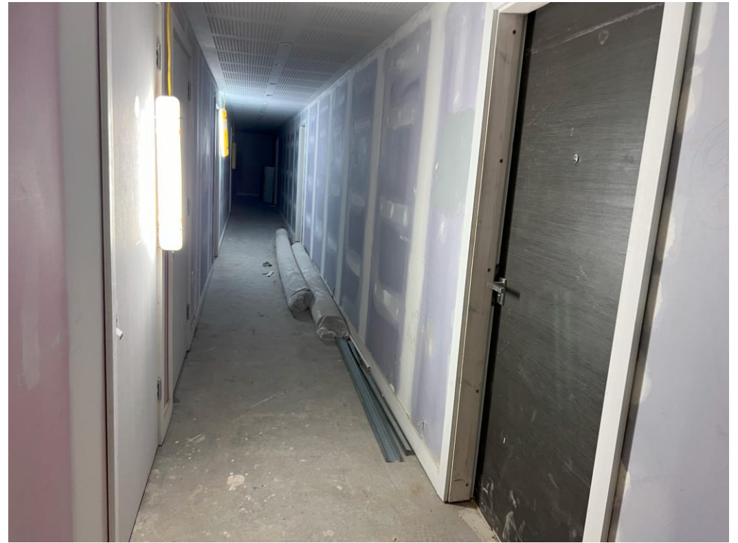
Level 6 – Apartment doors installed
