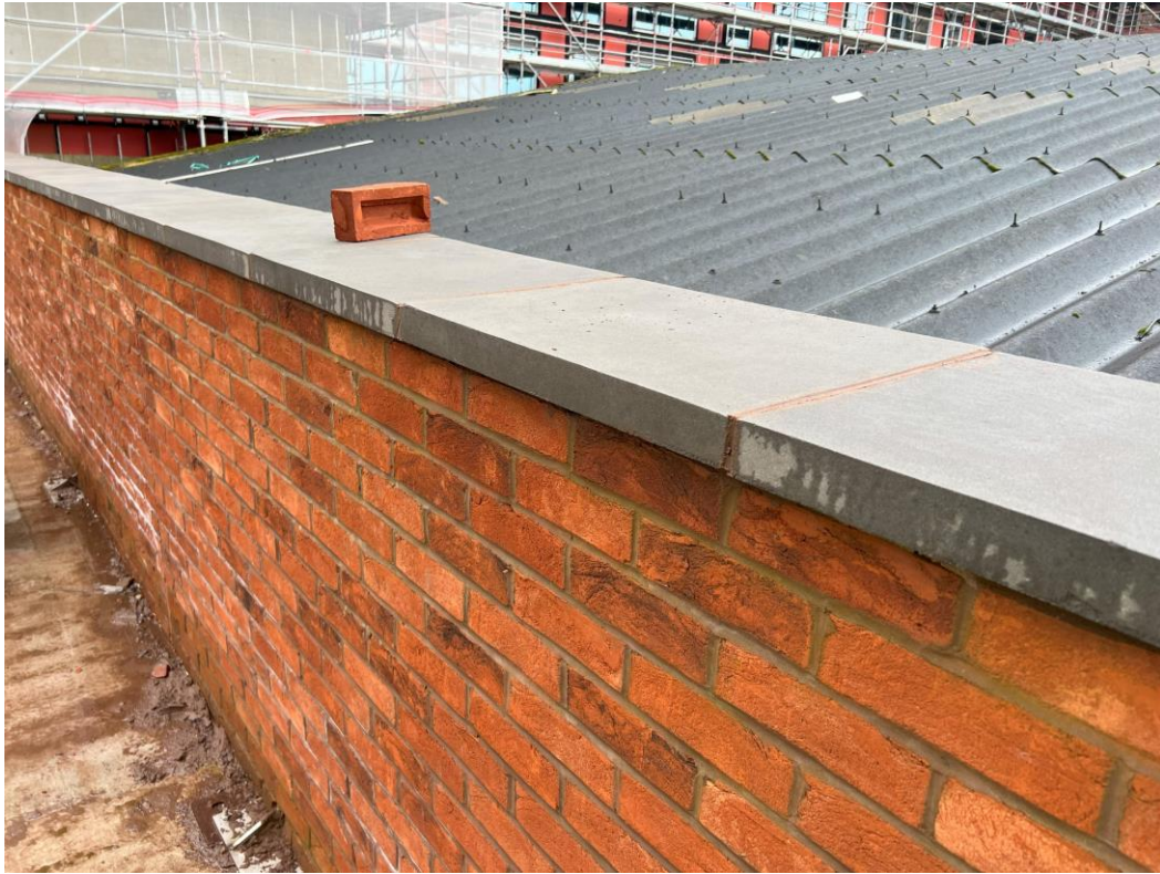
Coping stones installed
