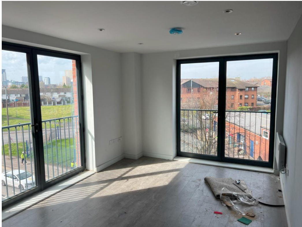
Level 5 – Laminate installed
