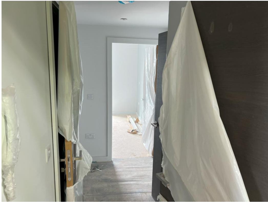
Level 7 – Doors installed
