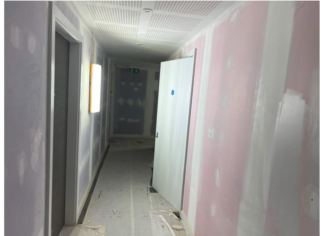
Level 3 – Corridor walls tape & jointed
