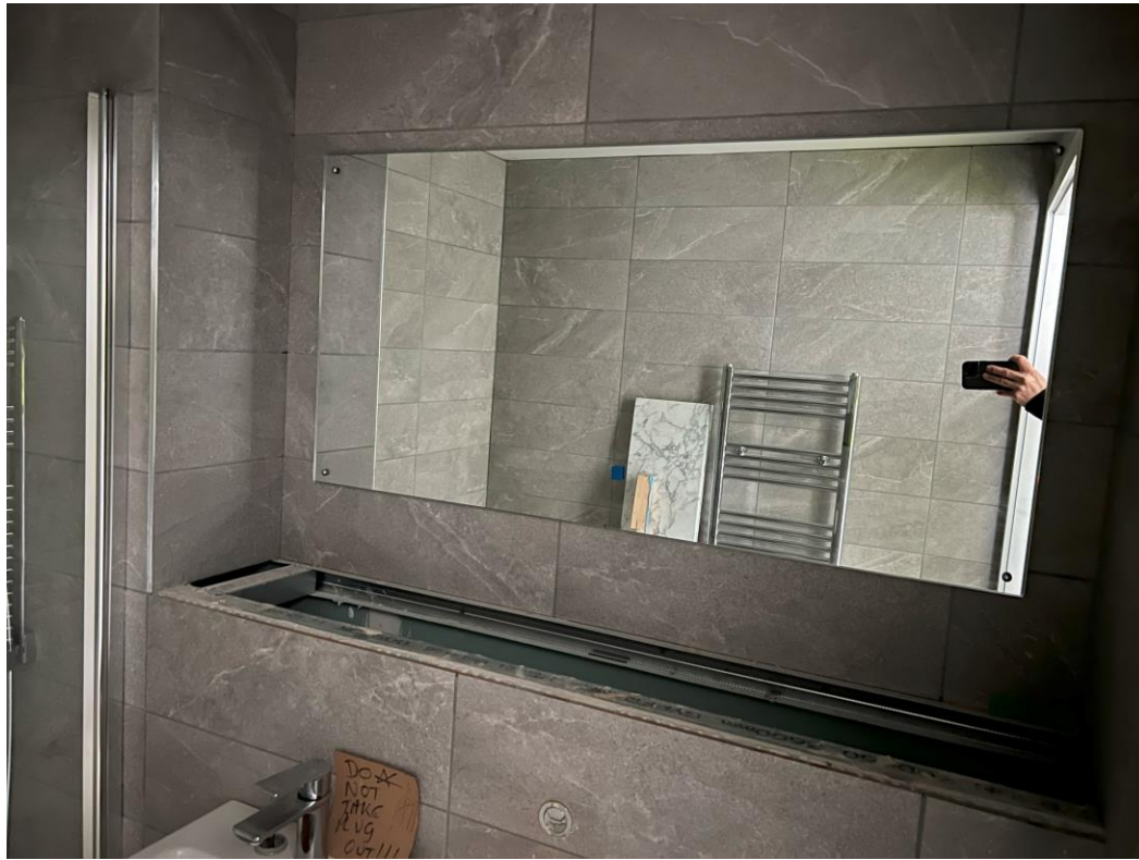
Level 5 – Bathroom mirror installed
