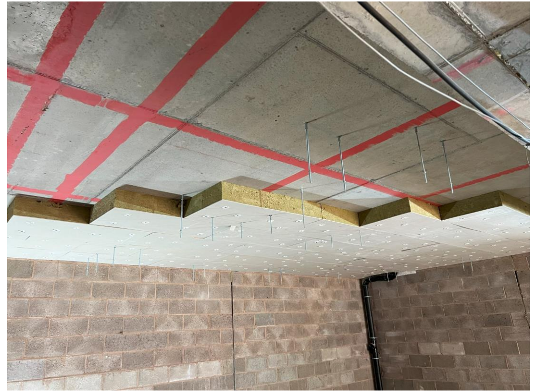
Ground Floor –Soffit insulation on-going
