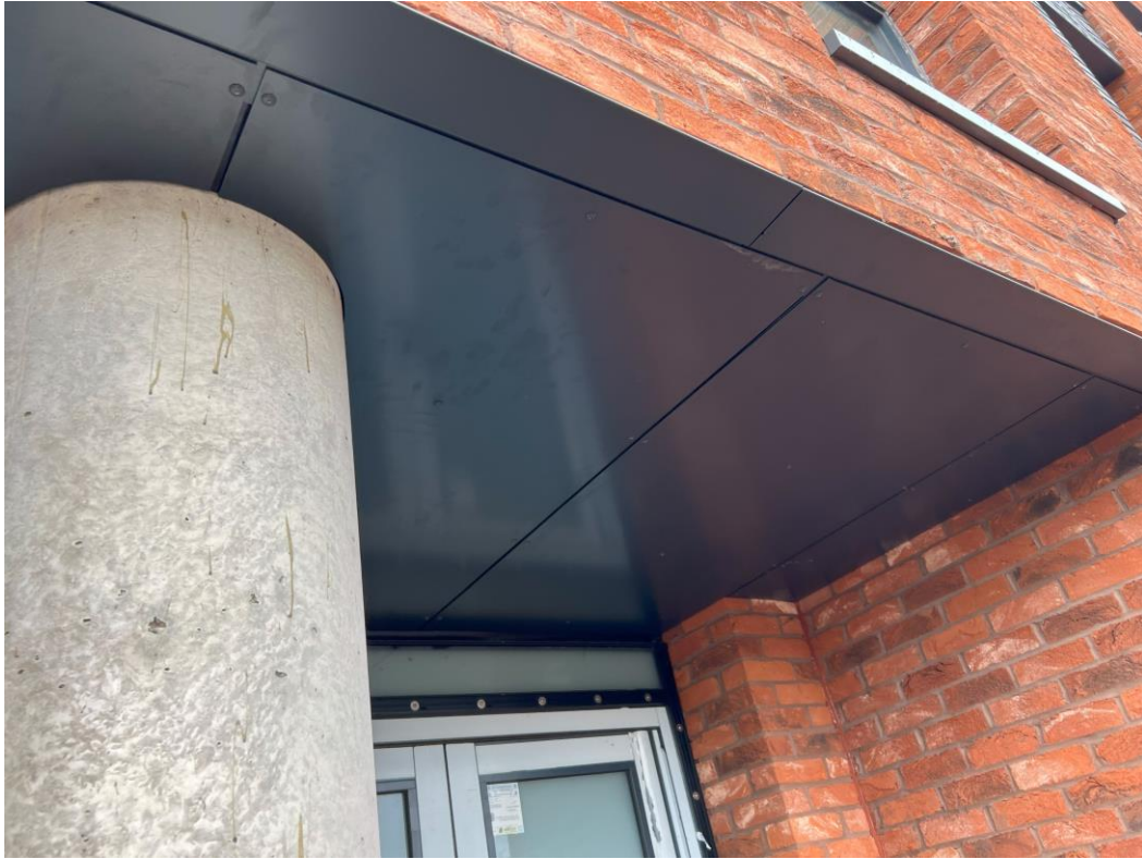
Block A – Soffit cladding installed
