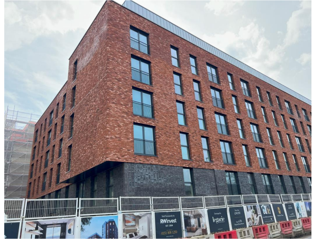
Block B – Viewed from Ordsall Lane
