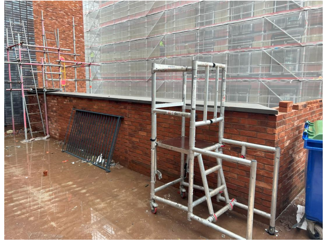
Coping stones installed
