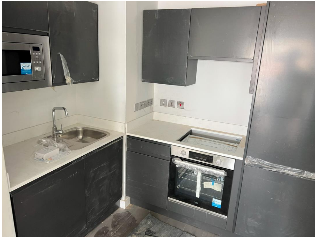
Level 5 – Kitchen complete
