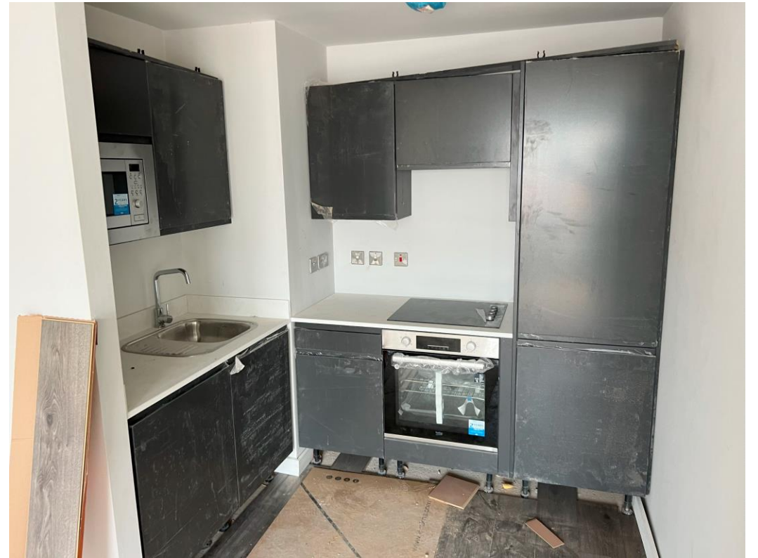
Level 6 – Kitchen installation complete
