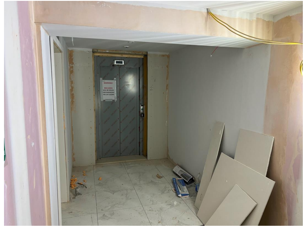
Level 4 - Lift lobby decoration
