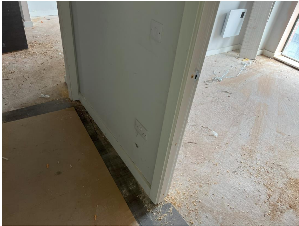
Level 6 – 2 nd fix joinery works on-going
