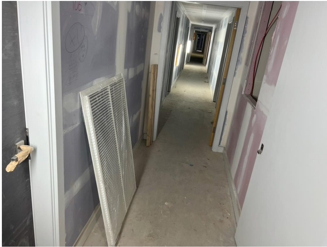
Level 6 – Louvre grills loaded for installation
