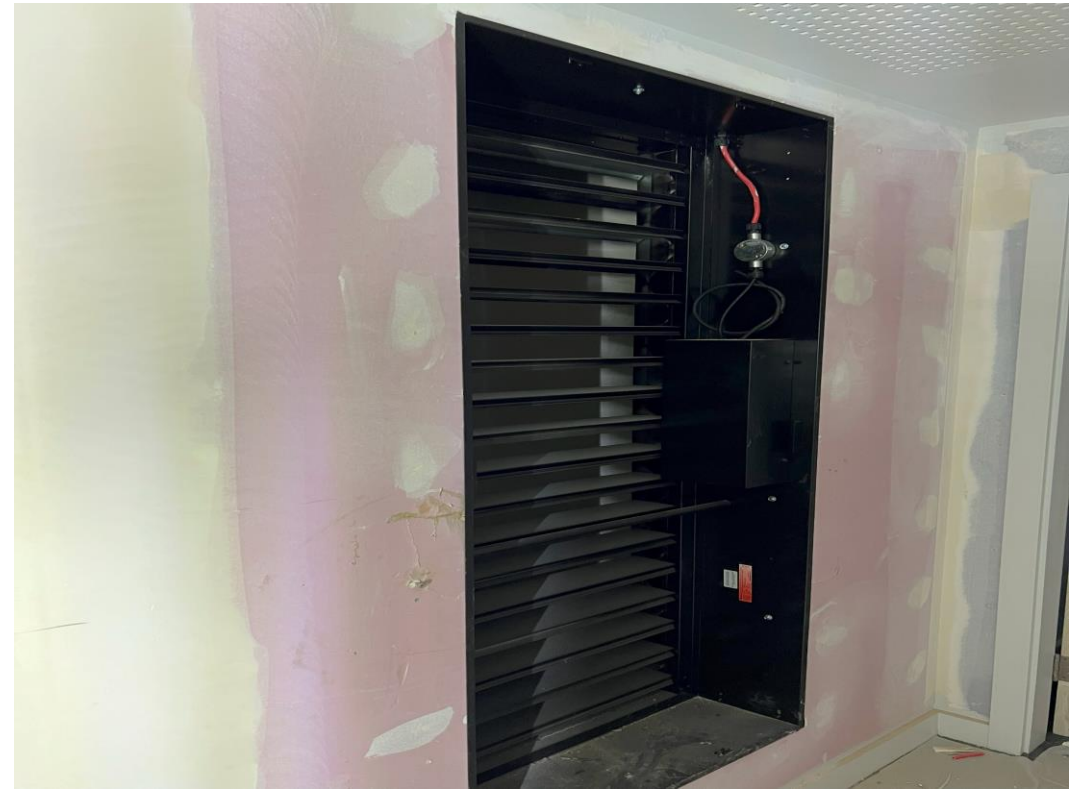
Level 6 – Louvre grills installed
