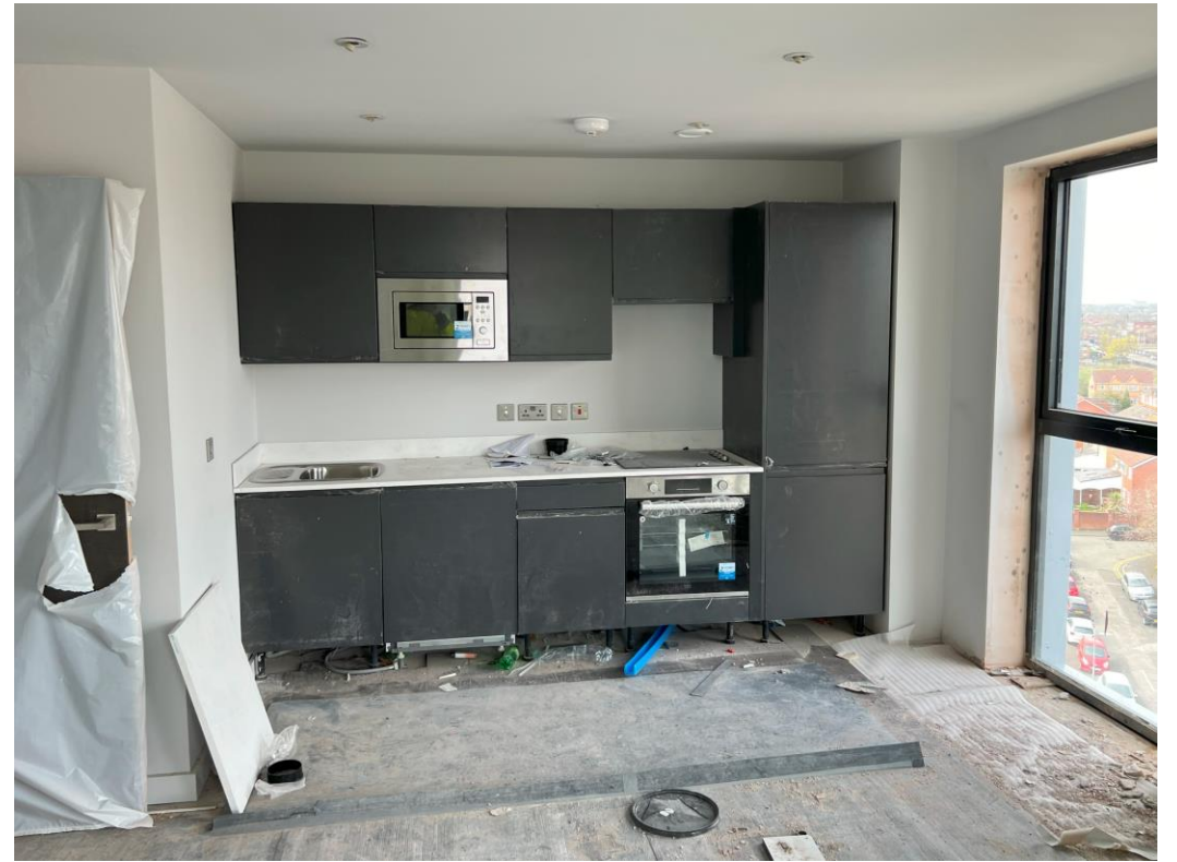
Level 8 – Appliances installed
