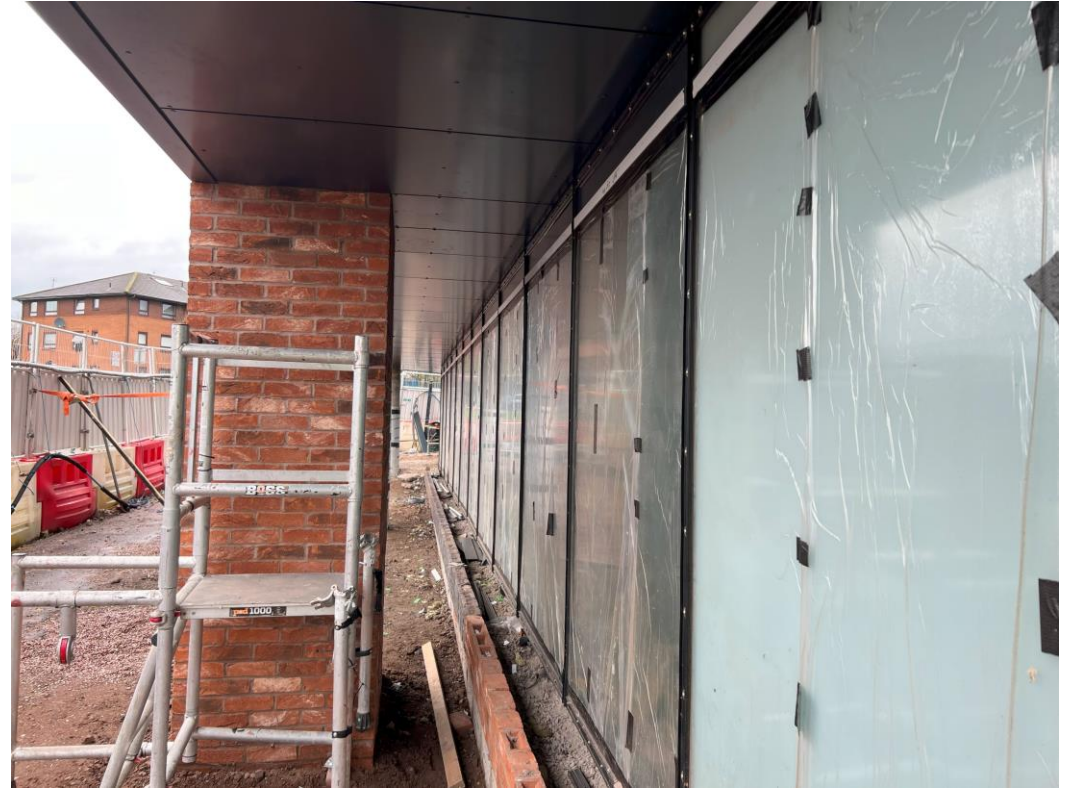
Block A – Soffit cladding installed
