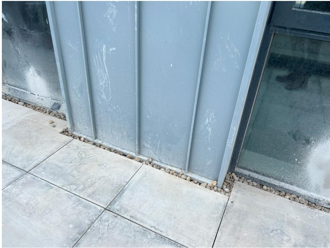
Block B concrete paving flags installed
