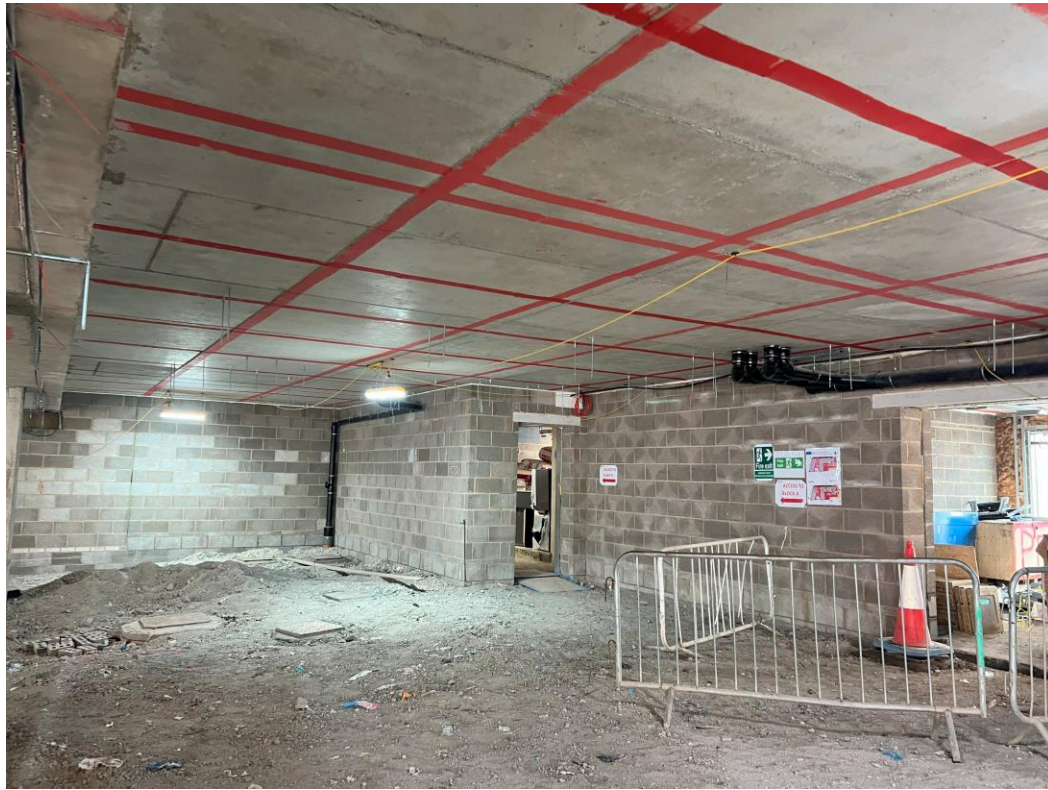
Ground Floor - General site activity
