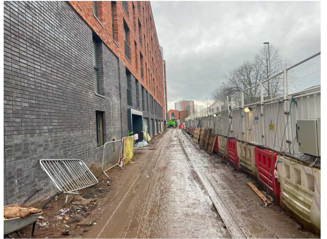
Block B – Viewed from Site Compound
