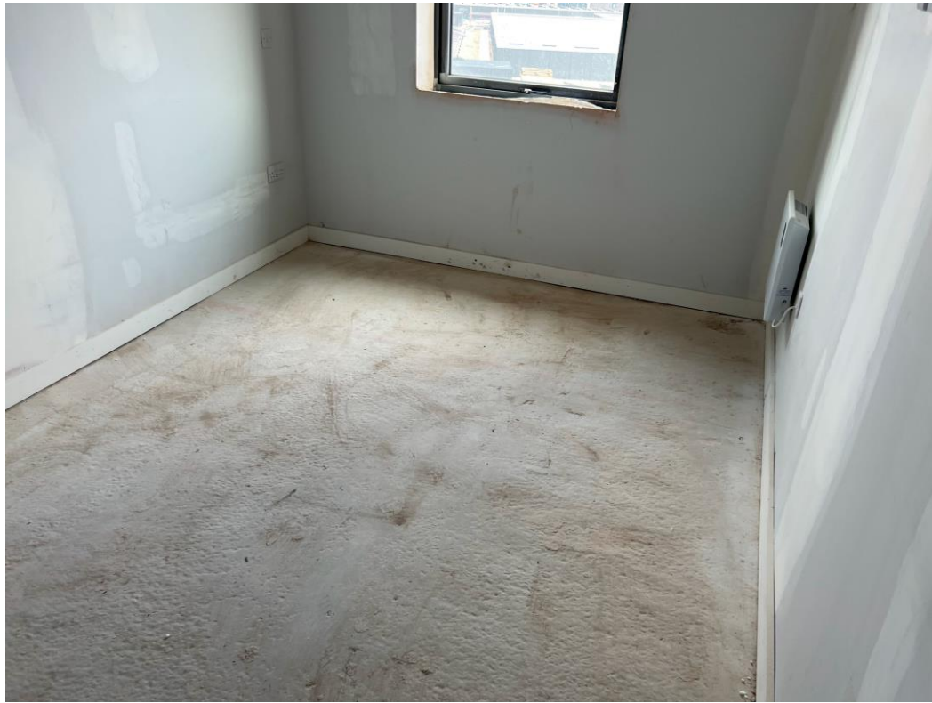
Level 8 – 2 nd fix joinery
