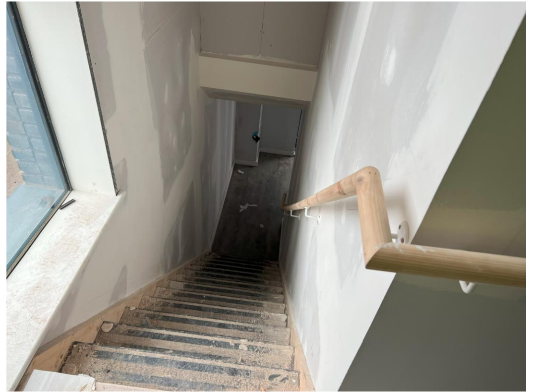
Ground Floor – Stair handrails installed
