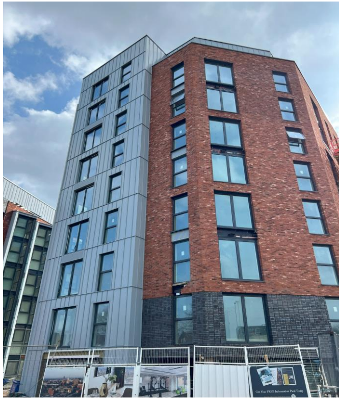
Ordsall Lane site view
