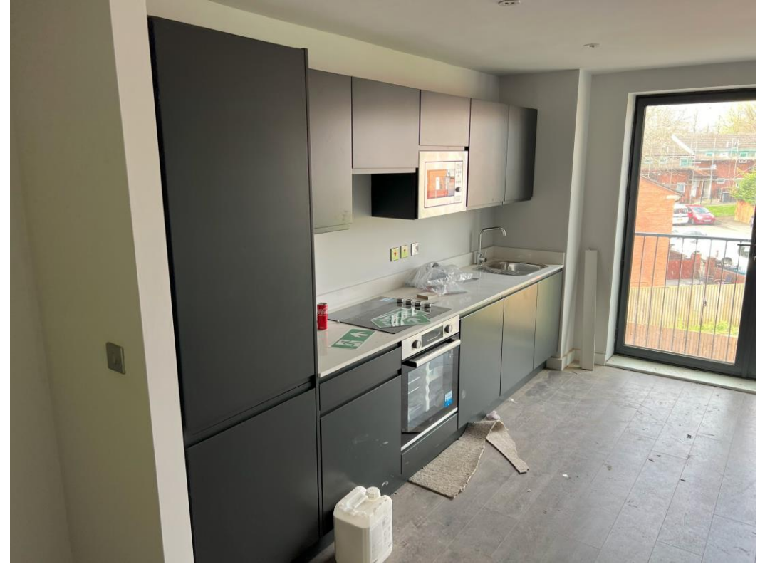
Level 3 – kitchen units & worktops installed
