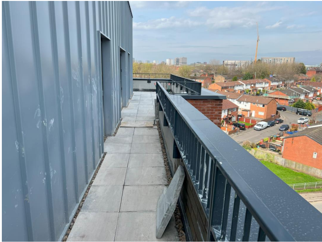
Block A Balustrade handrail
