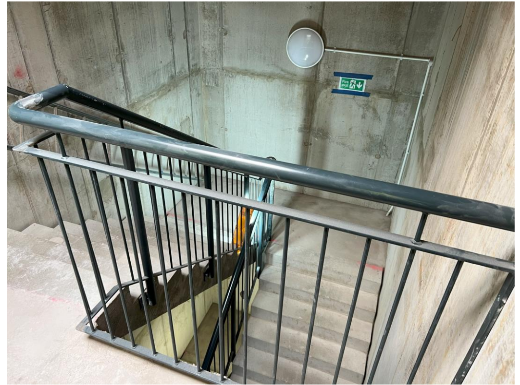
Level 6 - Stairwell balustrades
