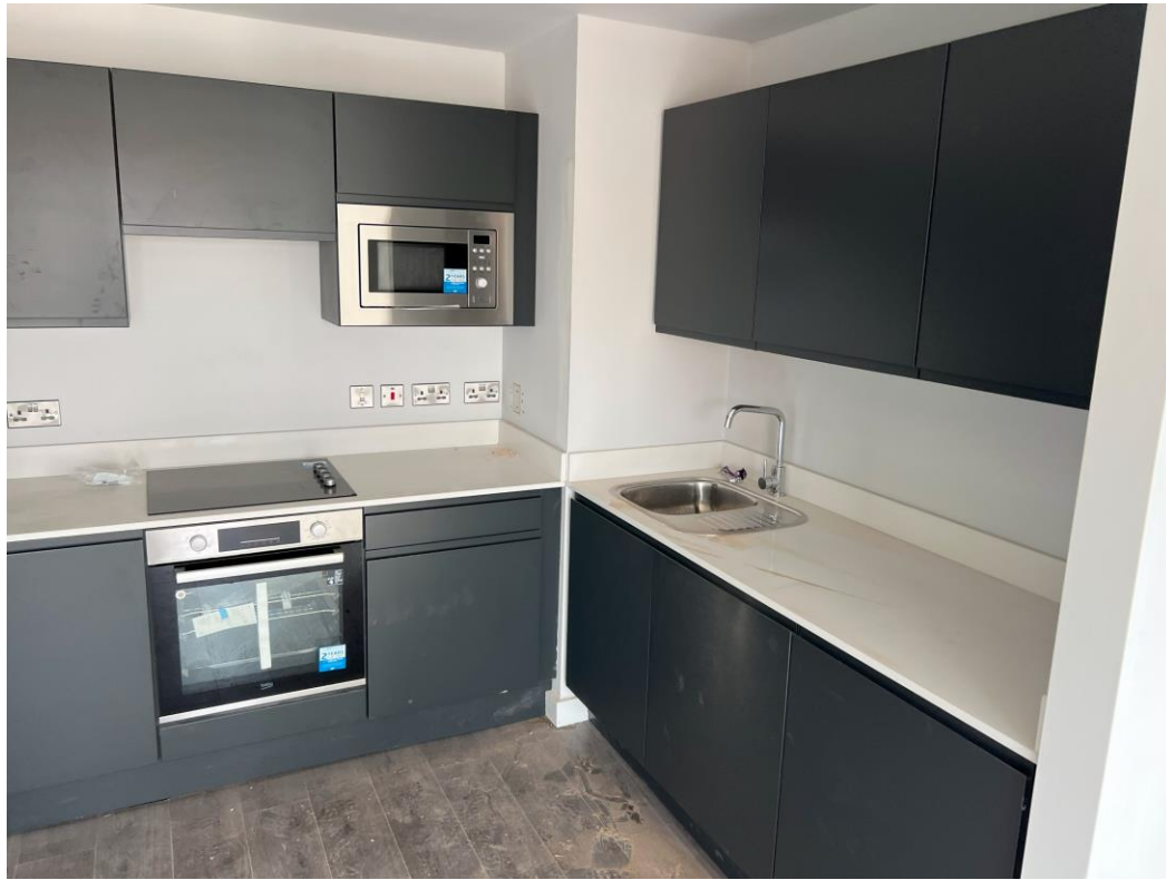
Level 5 – Kitchen units installed
