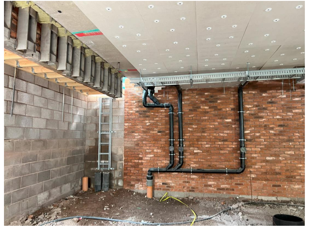
Ground Floor –Soffit insulation on-going
