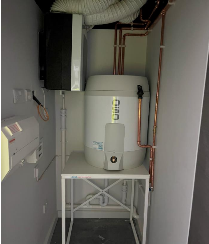
Level 3 – 2 nd fix mechanical & electrical
