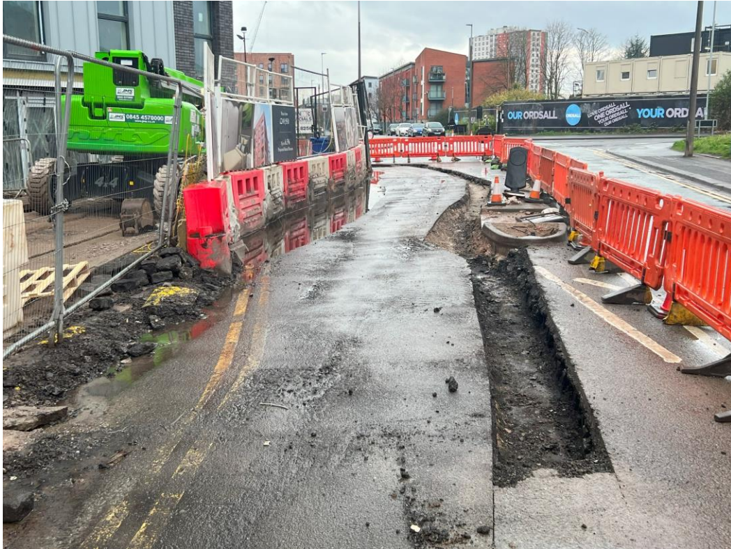
Ground works ongoing
