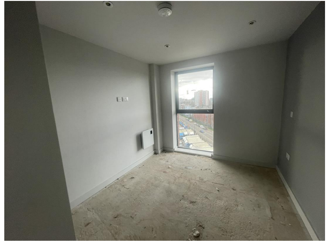
Level 7 – 2 nd fix joinery
