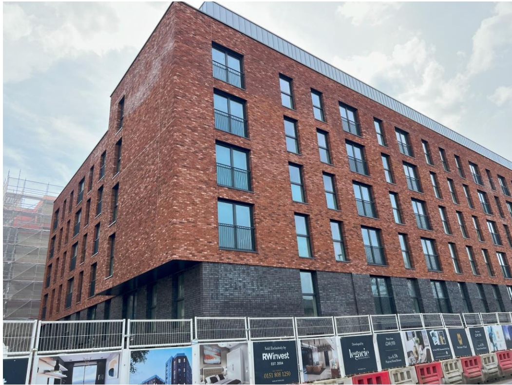
Ordsall Lane site view
