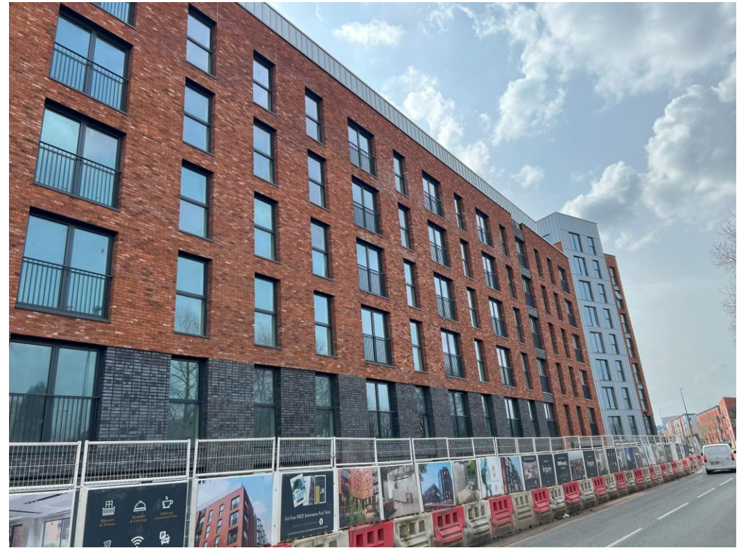
Ordsall Lane site view
