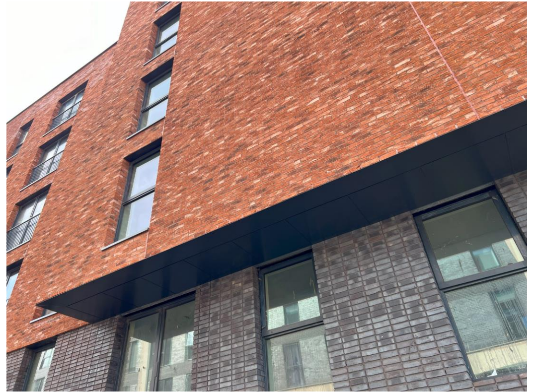
Ordsall Lane site view
