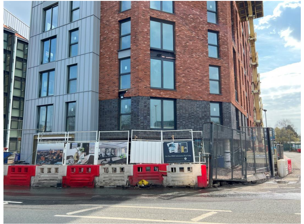
Ordsall Lane site view
