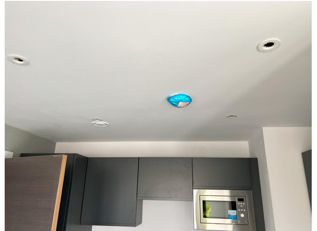
Level 5 – Kitchen smoke heads installed
