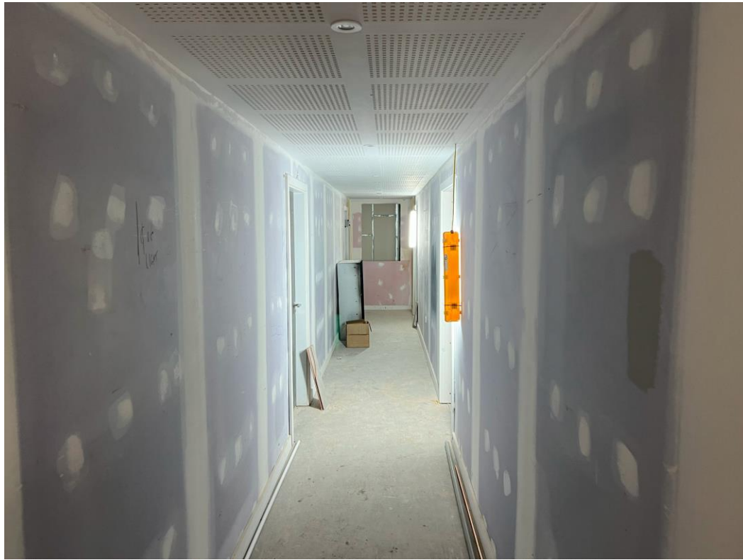
Level 6 – Circulation walls tape & jointed
