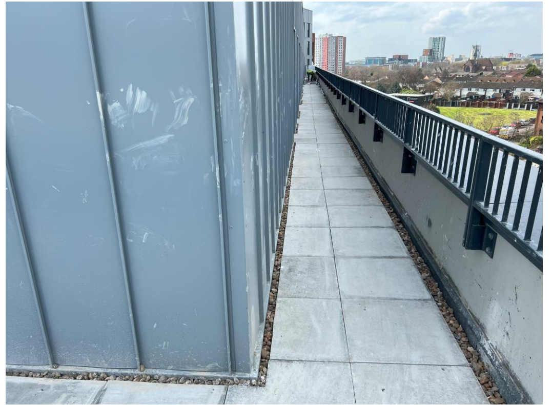
Block B concrete paving flags installed
