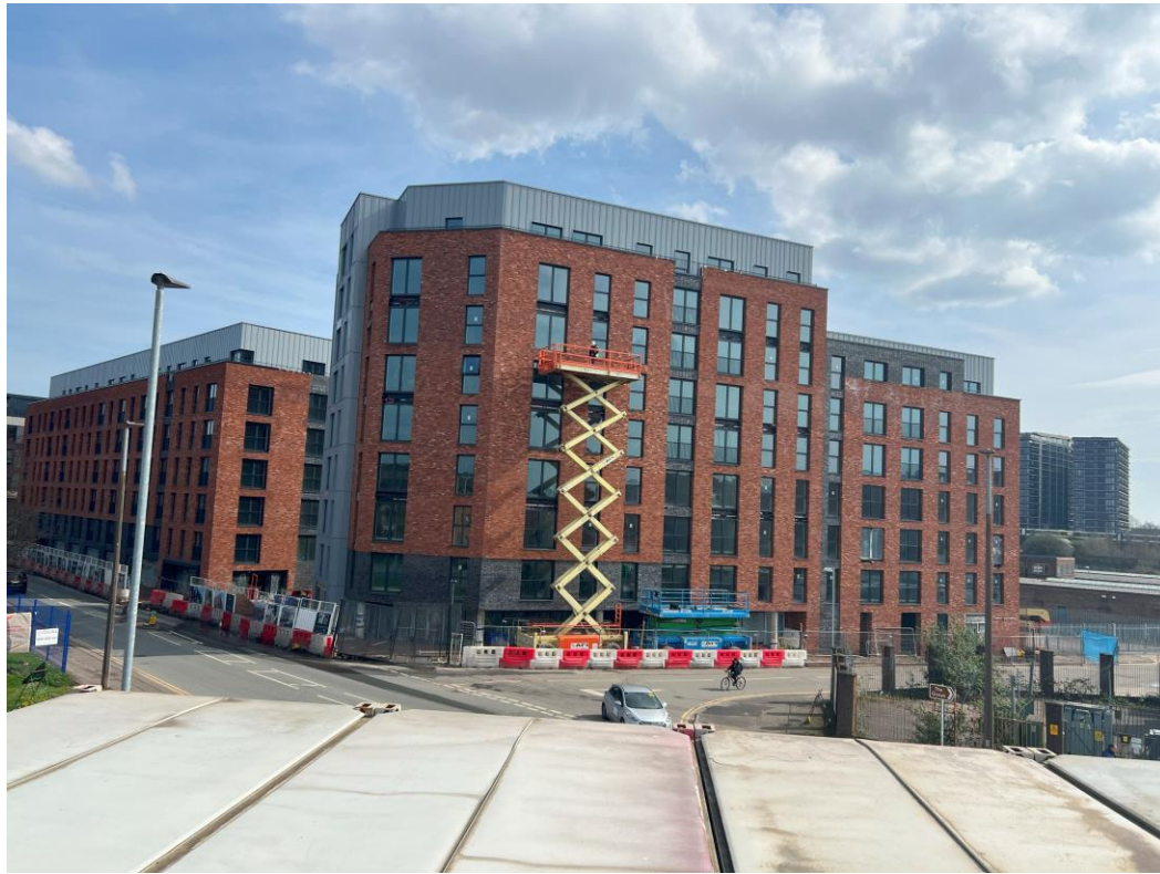
Ordsall Lane site view
