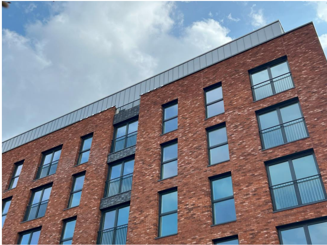
Ordsall Lane site view
