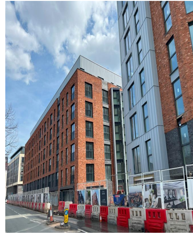
Ordsall Lane site view
