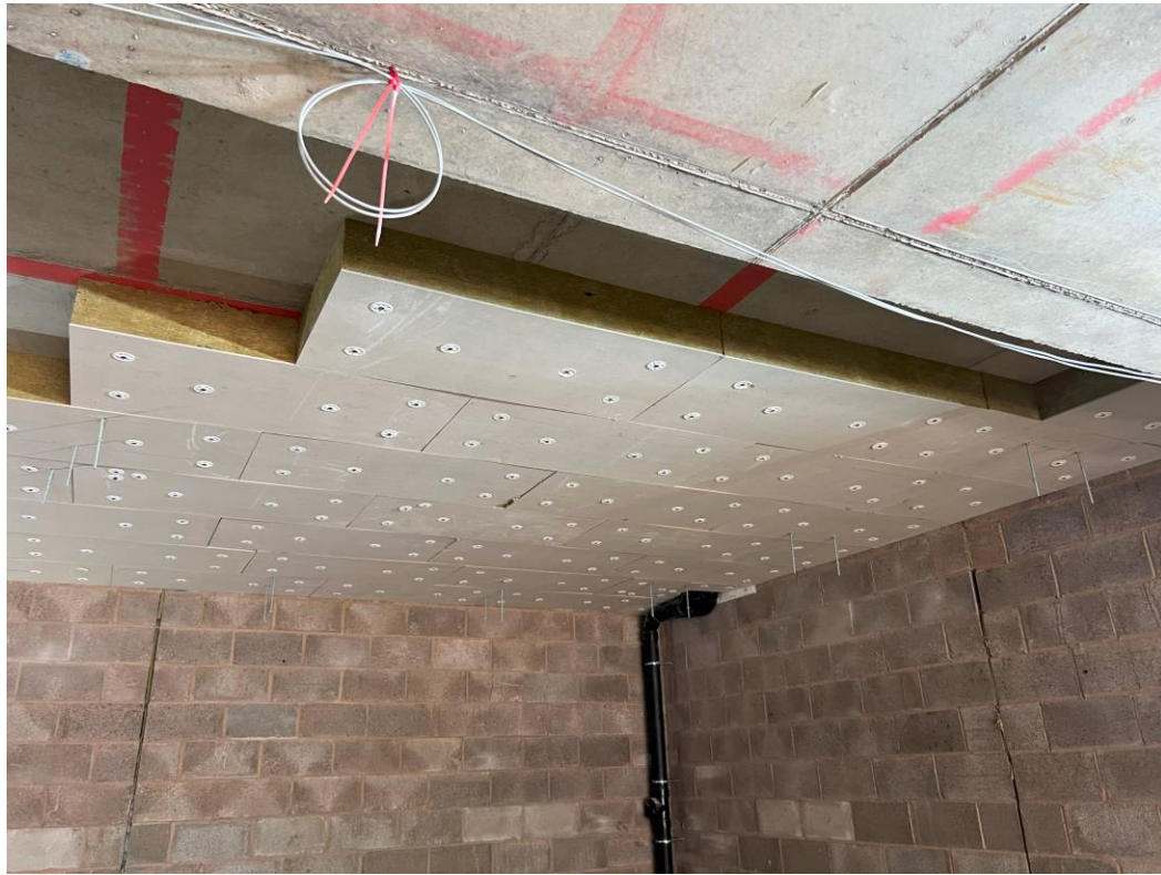
Ground Floor –Soffit insulation on-going
