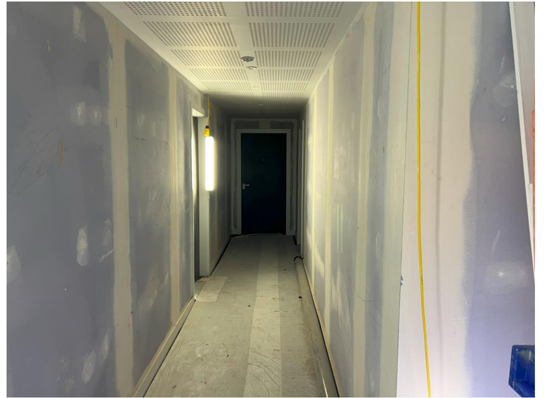
Level 6 – Acoustic ceiling decoration corridor
