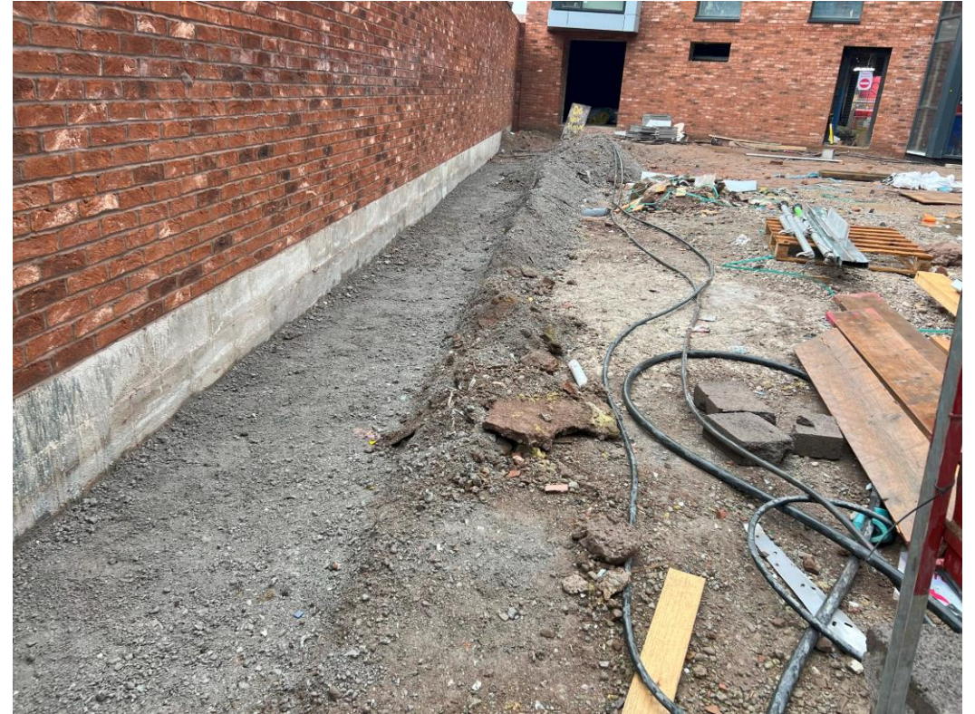
Ground works ongoing
