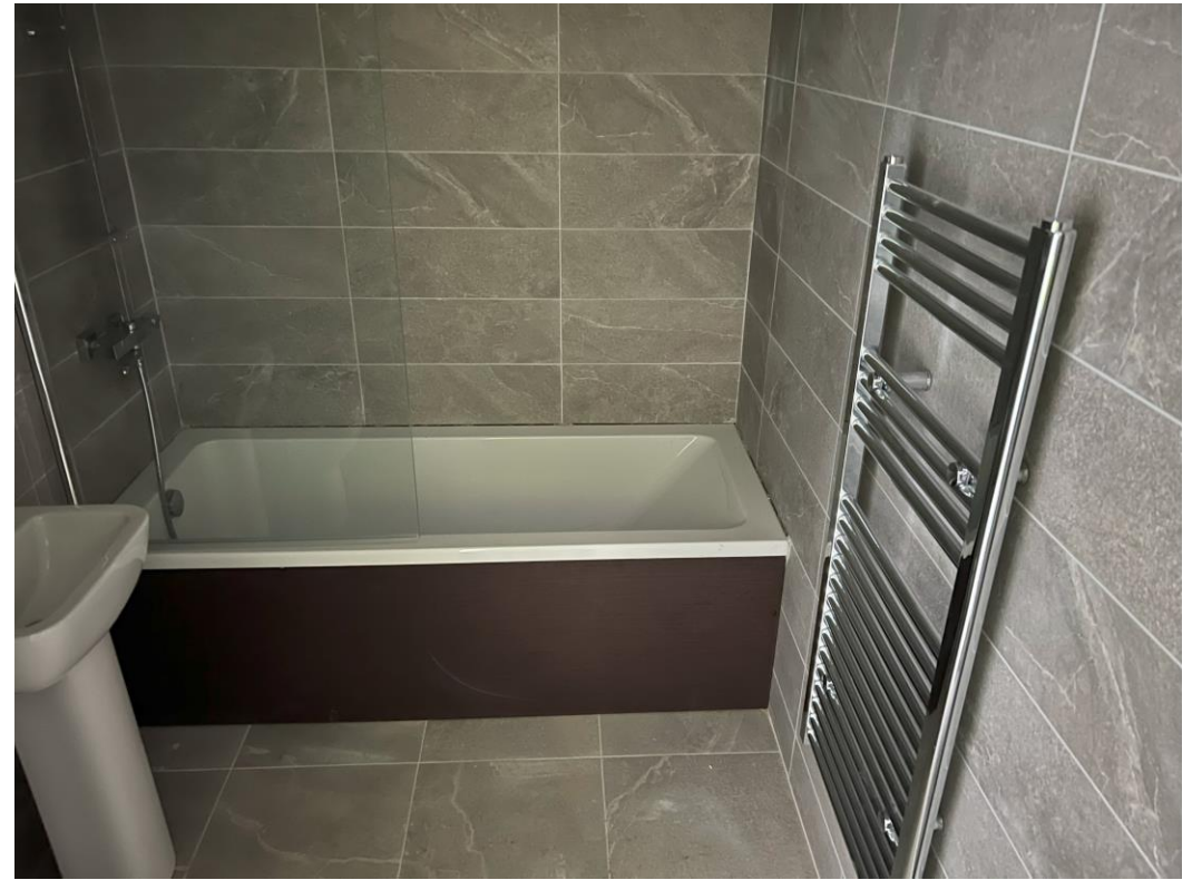
Level 4 – Heated towel radiator installed
