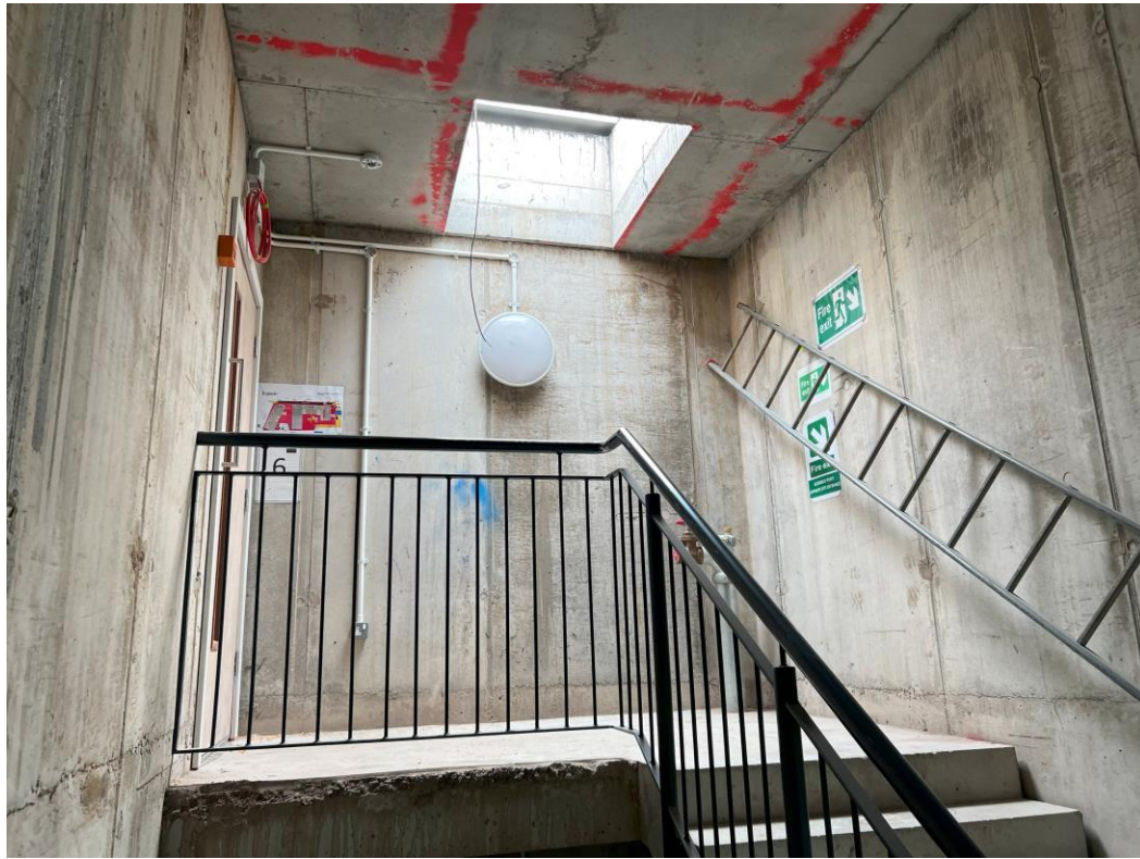
Level 6 - Stairwell balustrades
