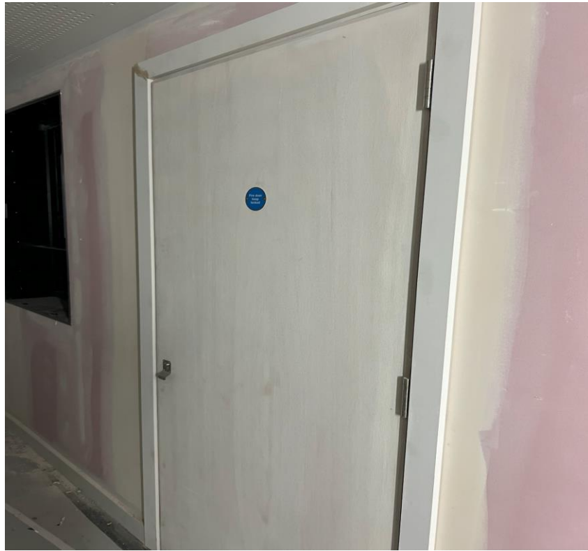
Level 6 – Service doors installed
