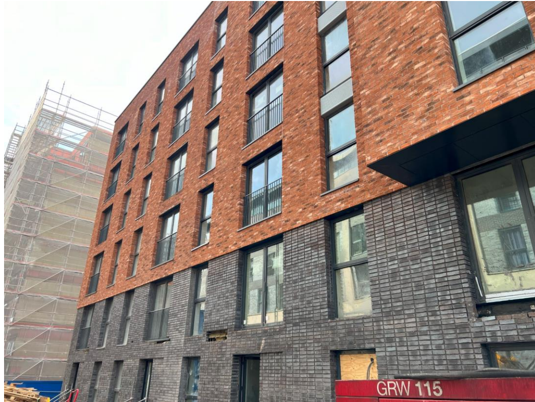
Block B – Viewed from Ordsall Lane
