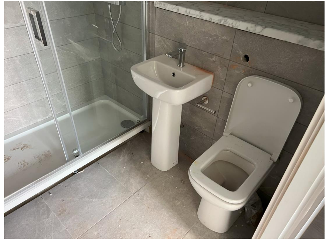
Level 5 - Bathroom sanitary items installed
