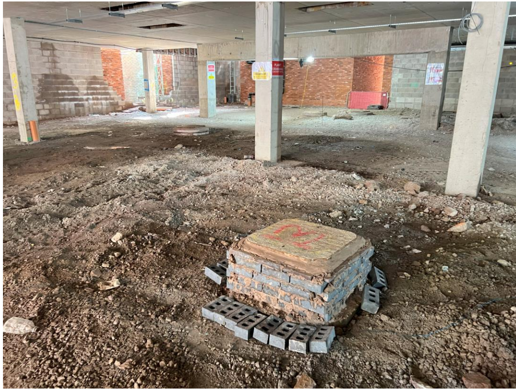
Ground Floor – Surface levelling commenced
