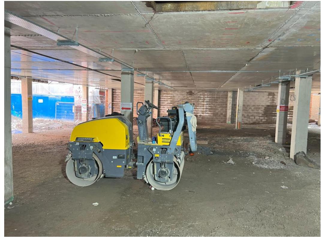
Ground Floor - Ground works ongoing
