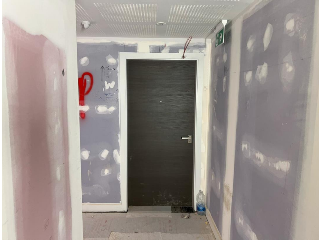
Level 3 – Apartment doors & ironmongery installed
