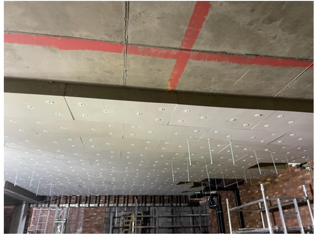
Podium – Soffit insulation installed
