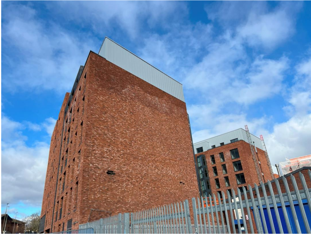
Block A – Viewed from Worrall Street
