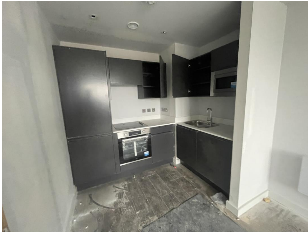
Level 6 – Kitchen units & worktops installed
