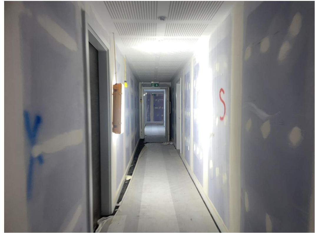
Level 6 – Corridor carpet
