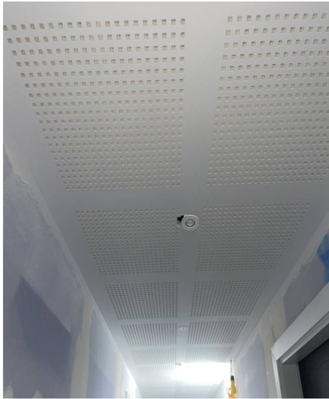
Level 6 – Acoustic ceiling decoration corridor
