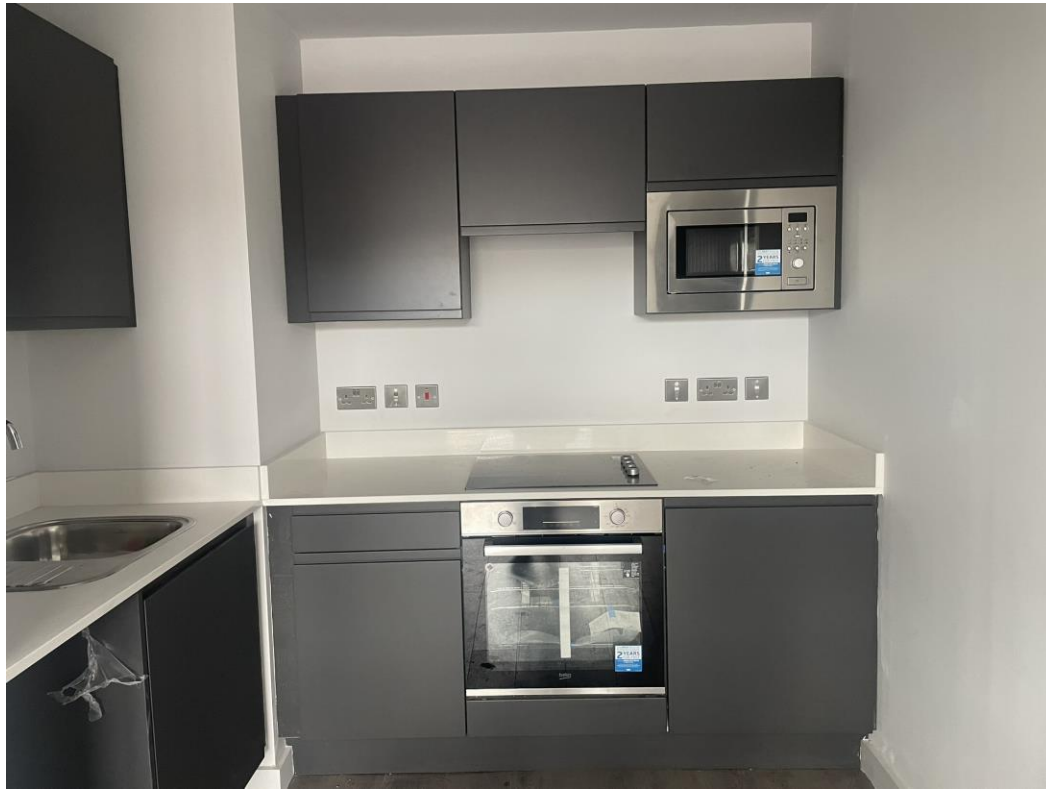
Level 6 – Kitchen installation complete
