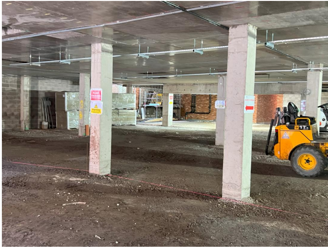
Ground Floor – Surface levelling commenced
