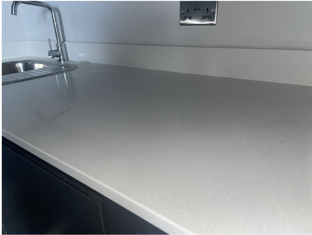
Level 6 – Worktops installed
