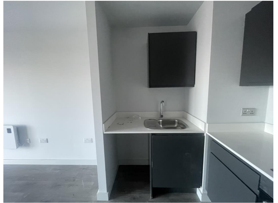
Level 4 – kitchen units & worktop installed
