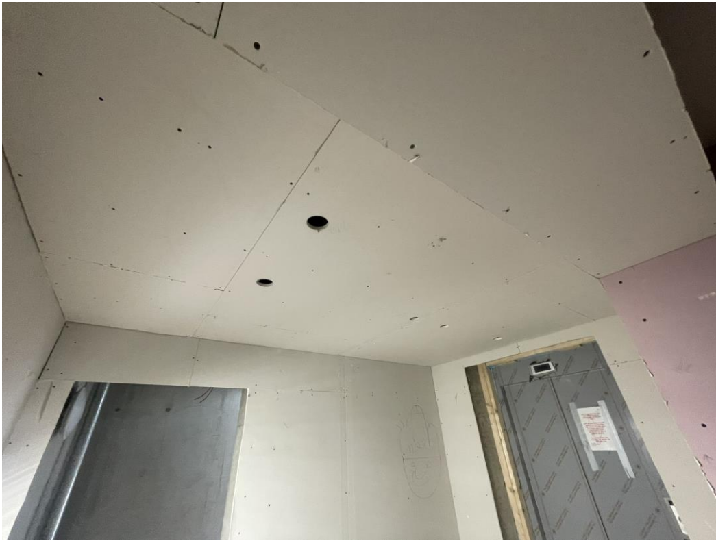
Level 6 – Lift lobby walls & ceilings boarded
