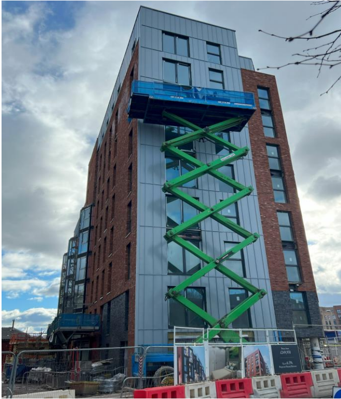
Ordsall Lane site view
