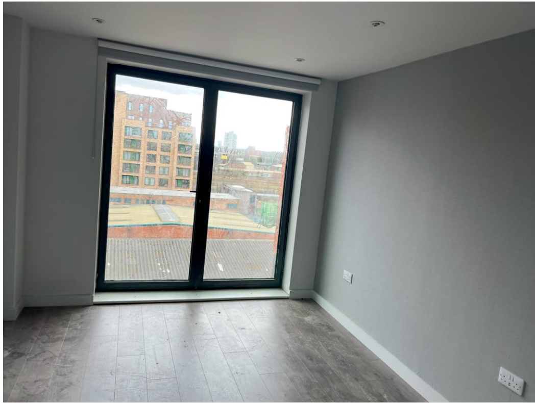
Level 8 – Laminate flooring installed
