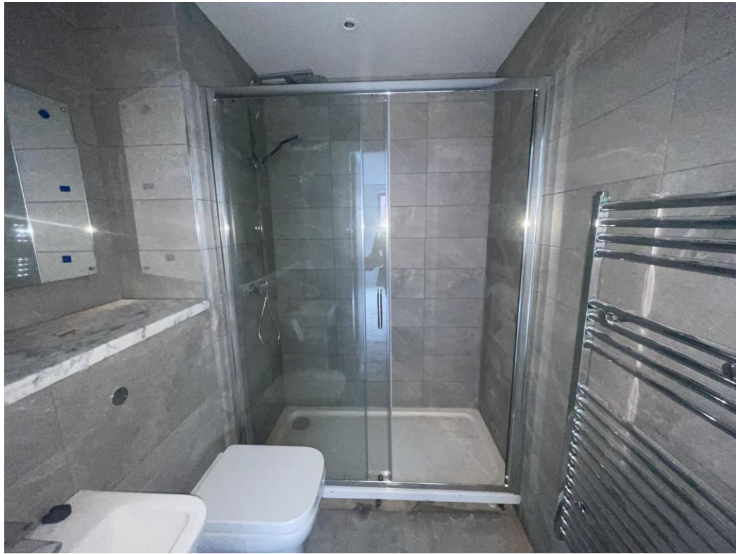
Level 2 – Shower screen installed
