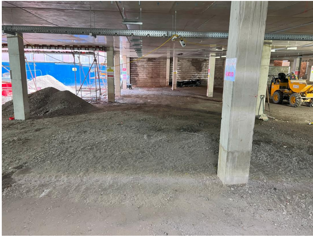
Ground Floor – Surface levelling commenced
