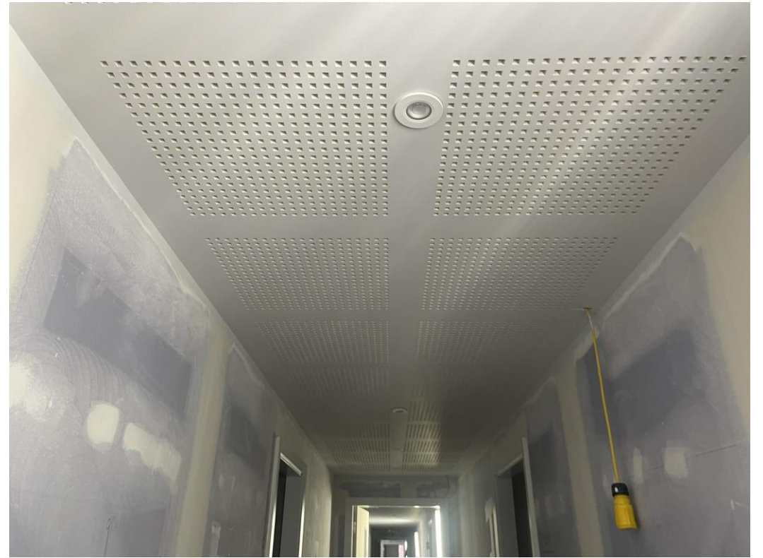
Level 6 – Acoustic ceiling decoration corridor
