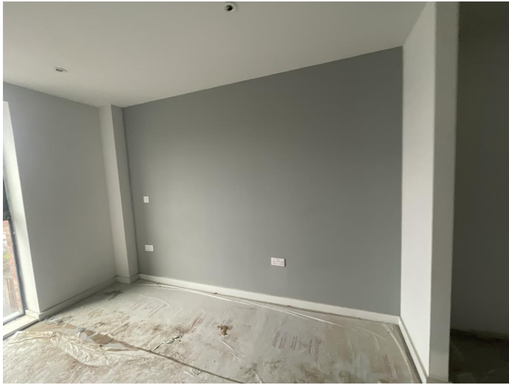
Level 5 – Feature wall finish
