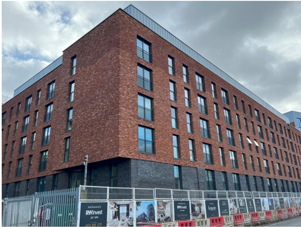
Ordsall Lane site view
