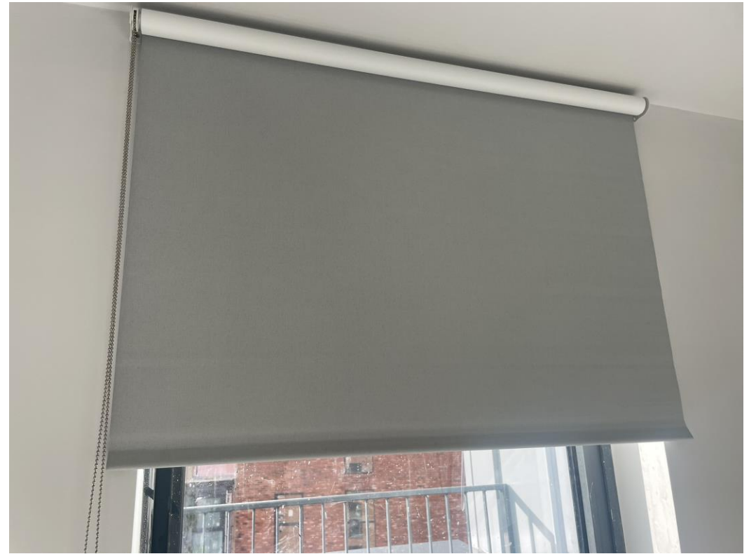
Level 6 – Blinds installed
