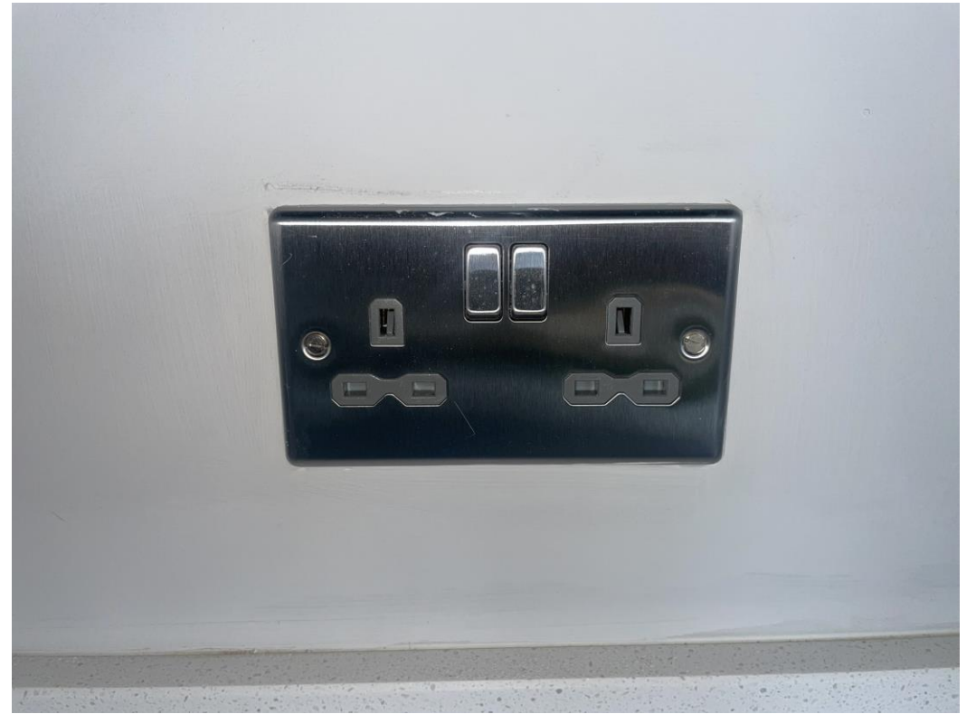
Level 6 – 2 nd fix electrical
