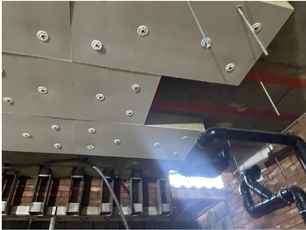
Podium – Soffit insulation installed
