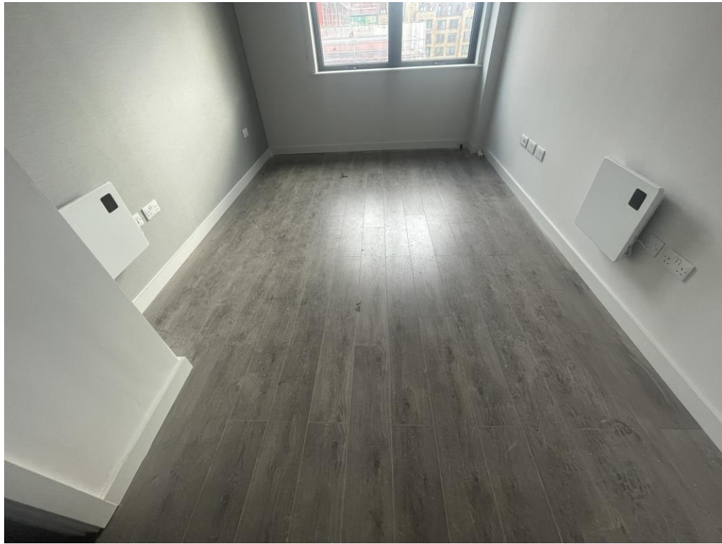
Level 5 – Laminate installed
