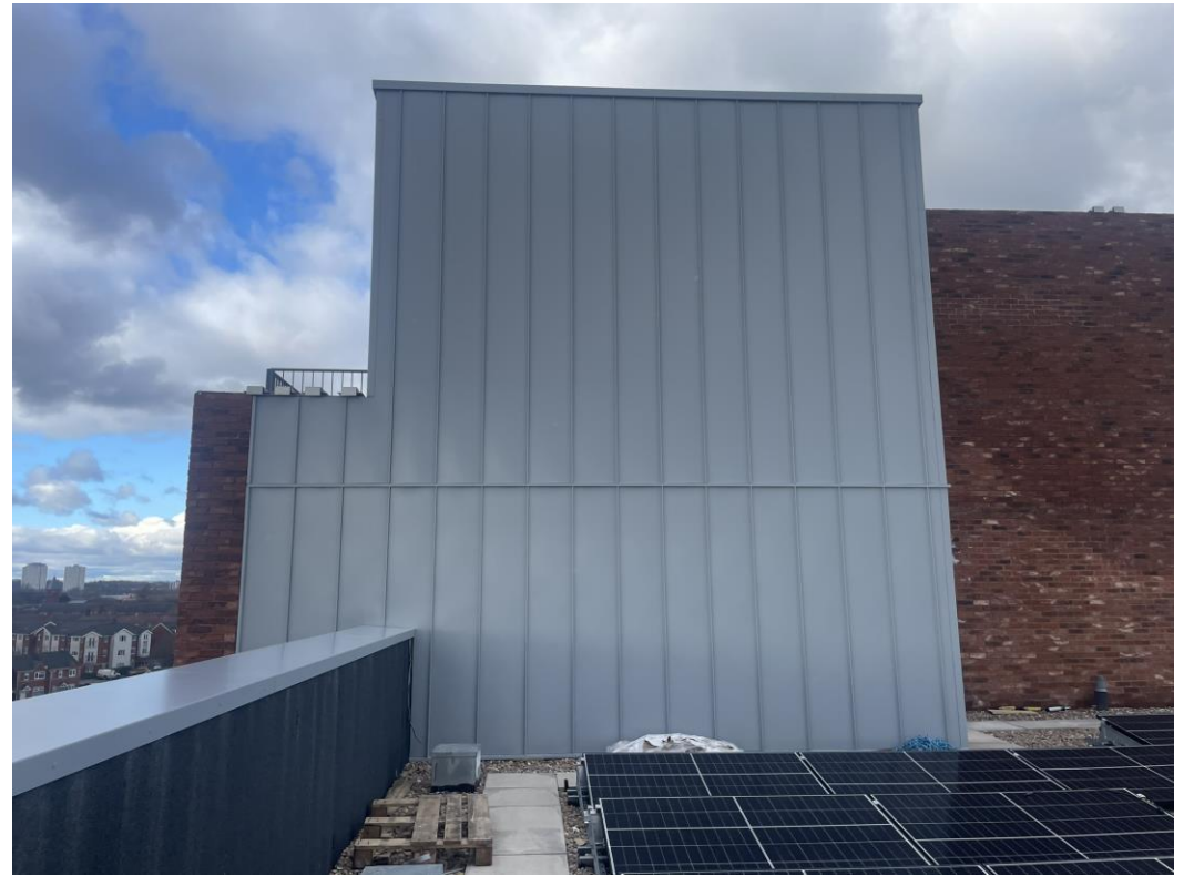
Block A Rainscreen cladding
