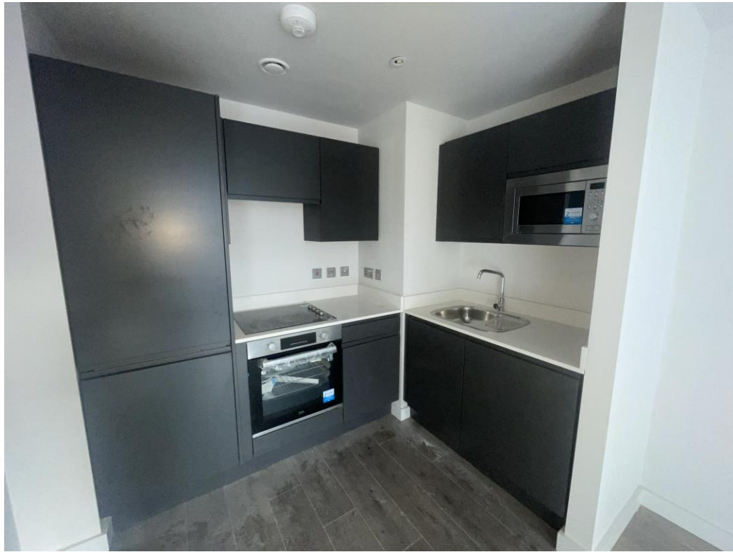
Level 5 – Kitchen units installed
