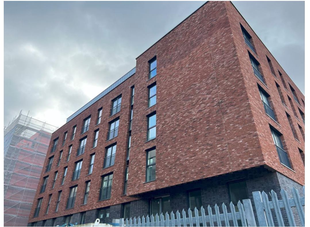
Ordsall Lane site view
