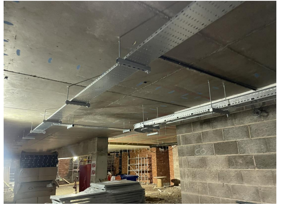
Ground Floor – Containment in place
