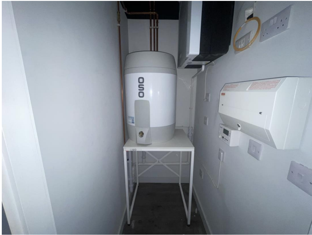
Level 6 – Second fix mechanical appliances
