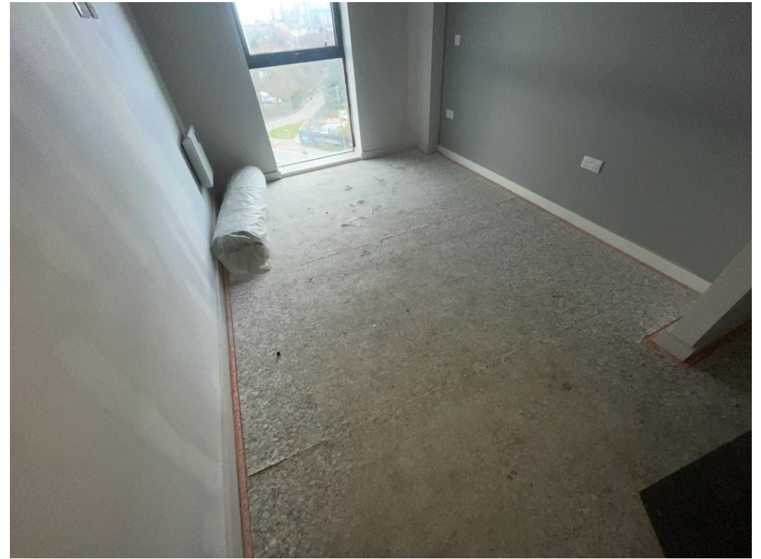
Level 6 – Underlay laid in preparation for carpet installation
