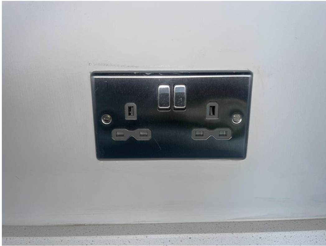
Level 1 – 2 nd fix electrical
