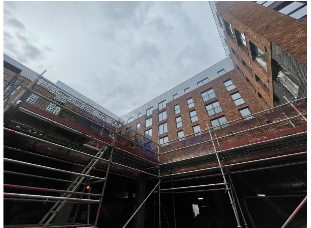
Podium site view
