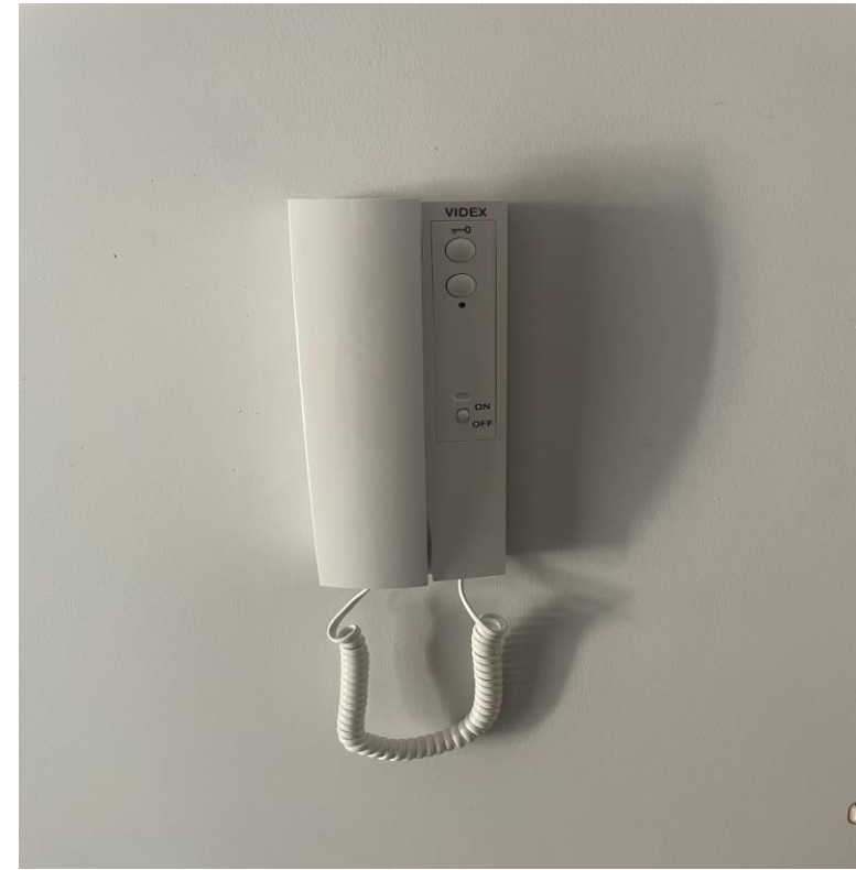
Level 6 – Telecom installed
