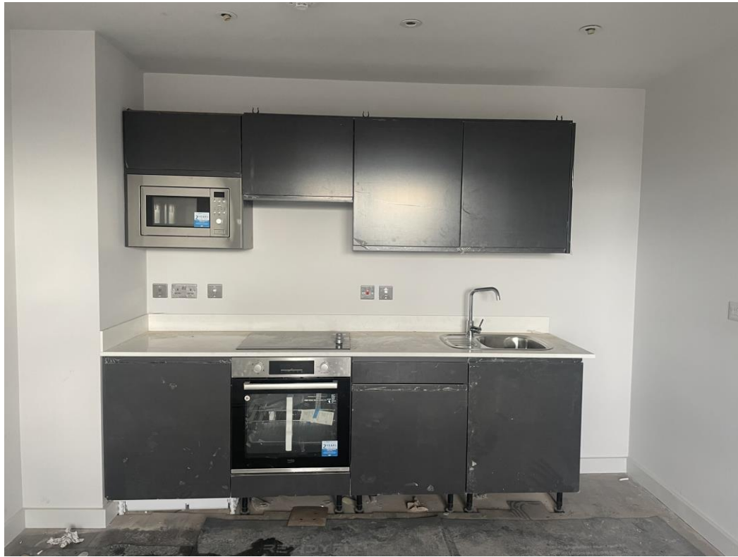
Level 8 – Kitchen units & worktops installed
