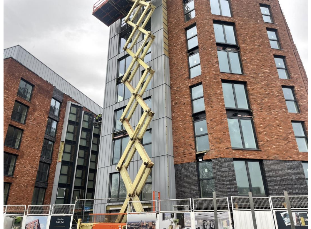
Ordsall Lane site view
