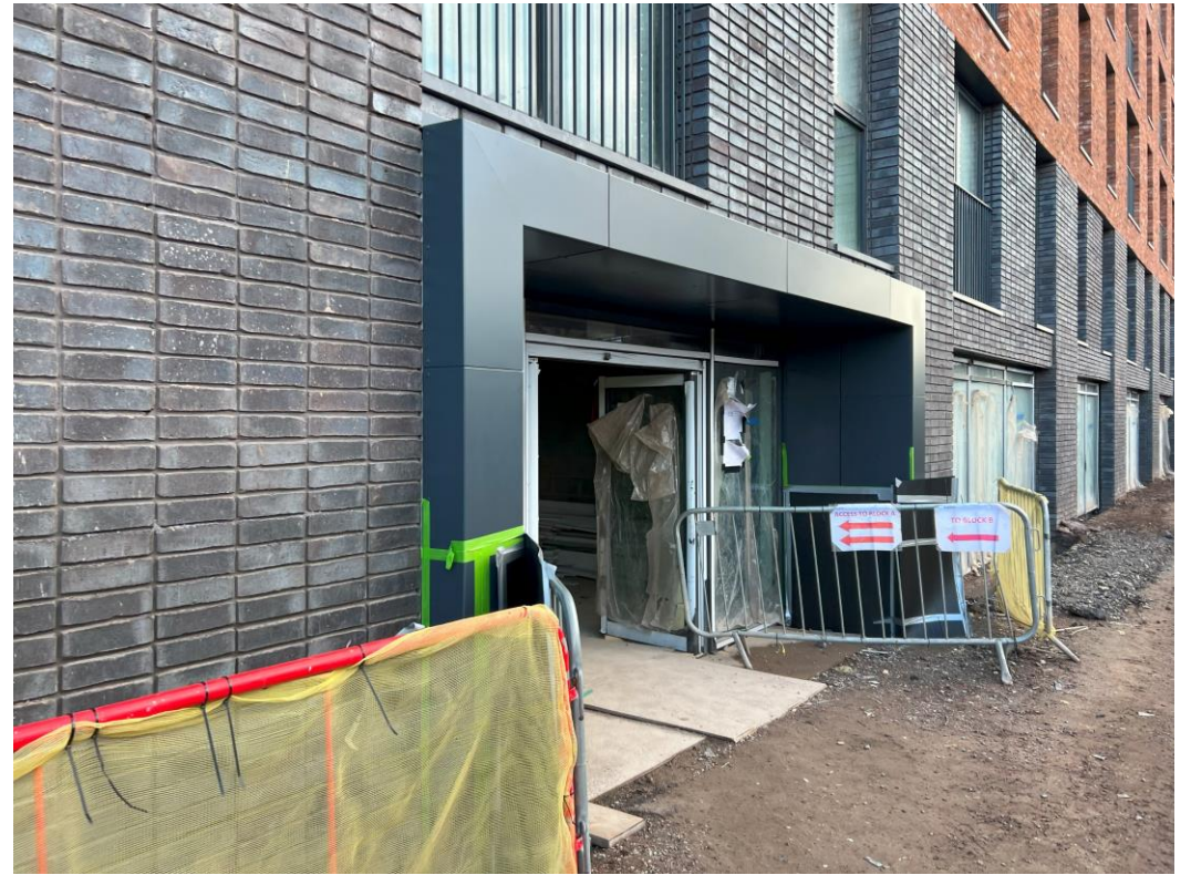
Cladding installed to entrance canopy
