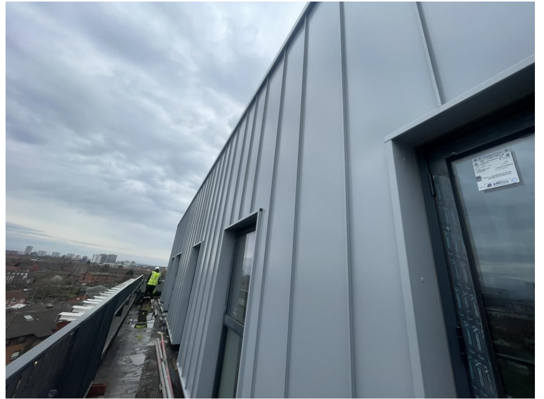
Block B rainscreen cladding
