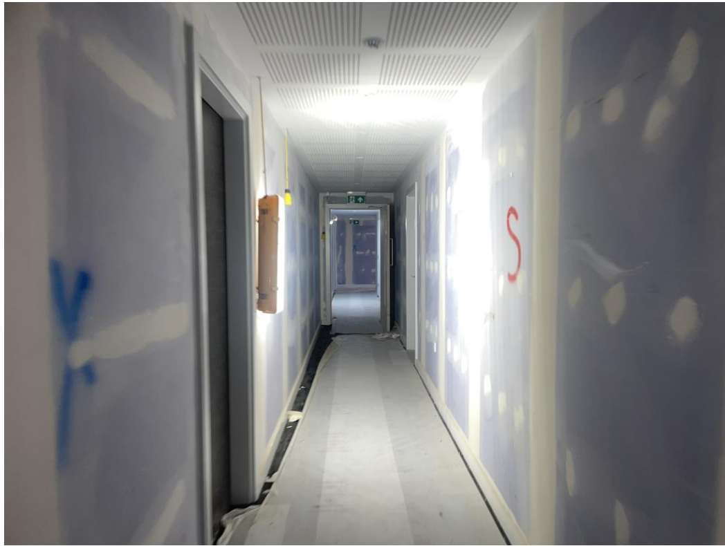
Level 5 – Corridor tape & jointing complete
