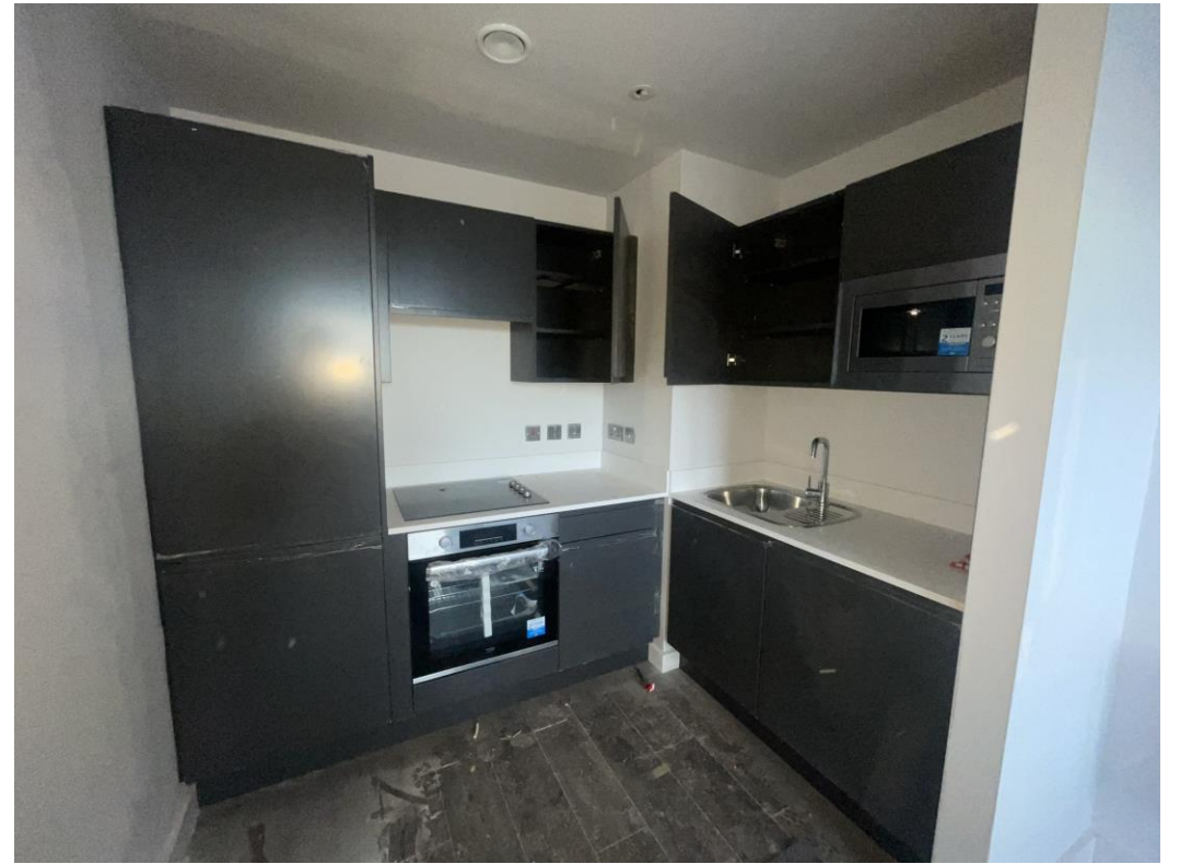
Level 8 – kitchen installed
