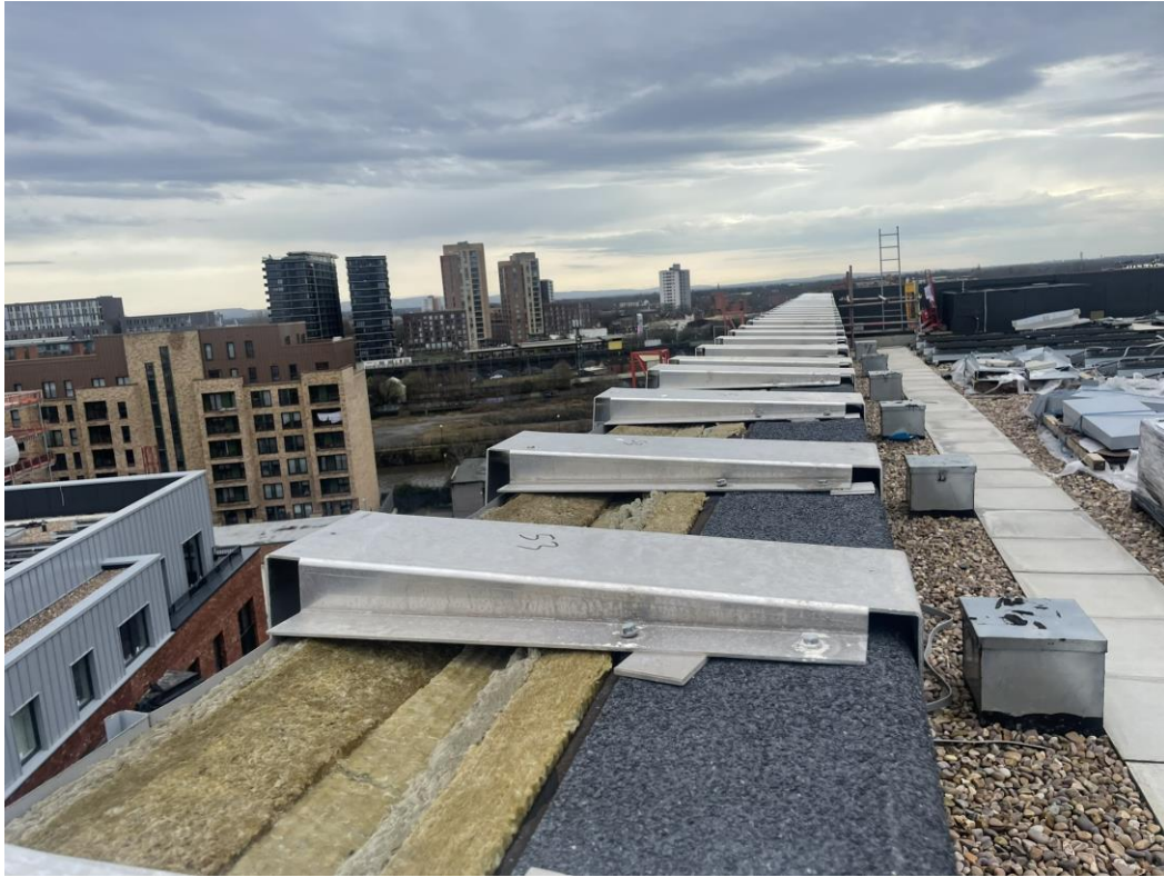
Block A – Parapet capping rails
