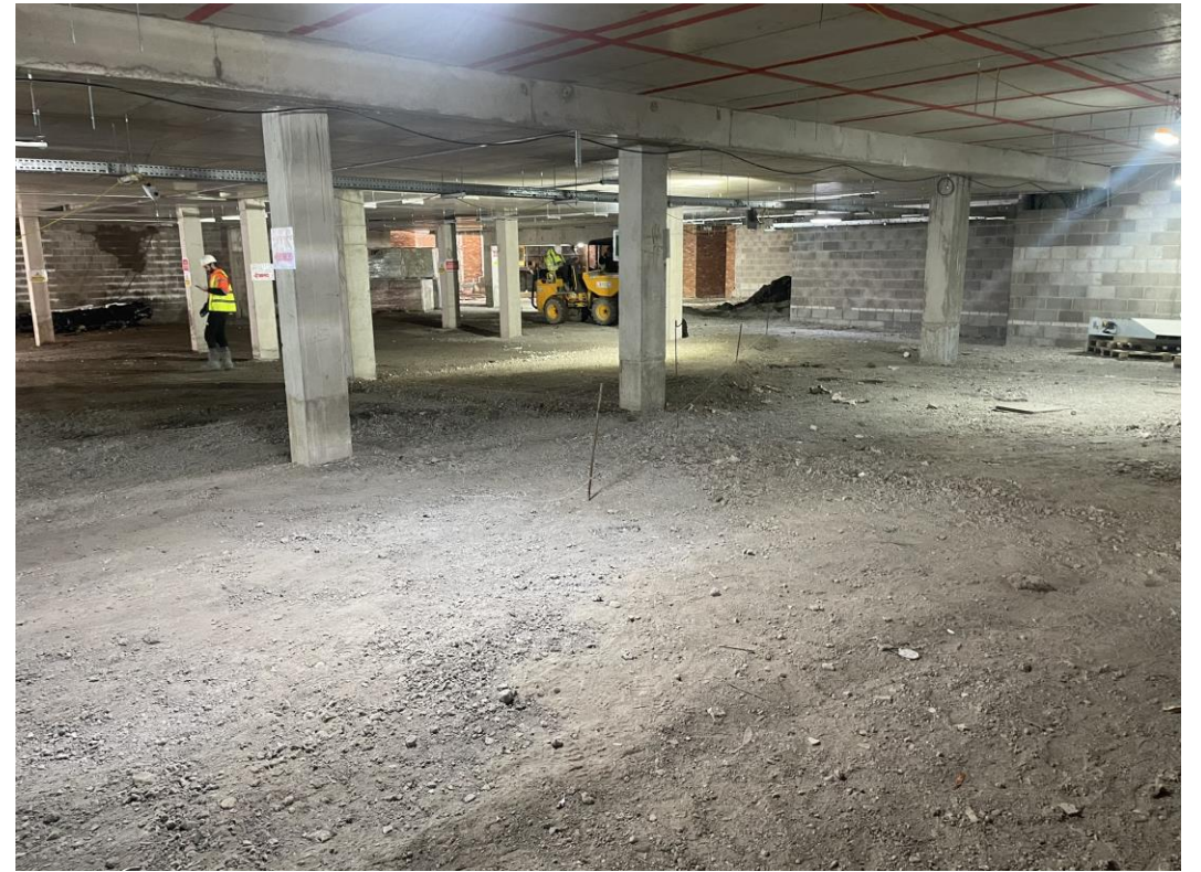
Ground Floor – Surface levelling commenced
