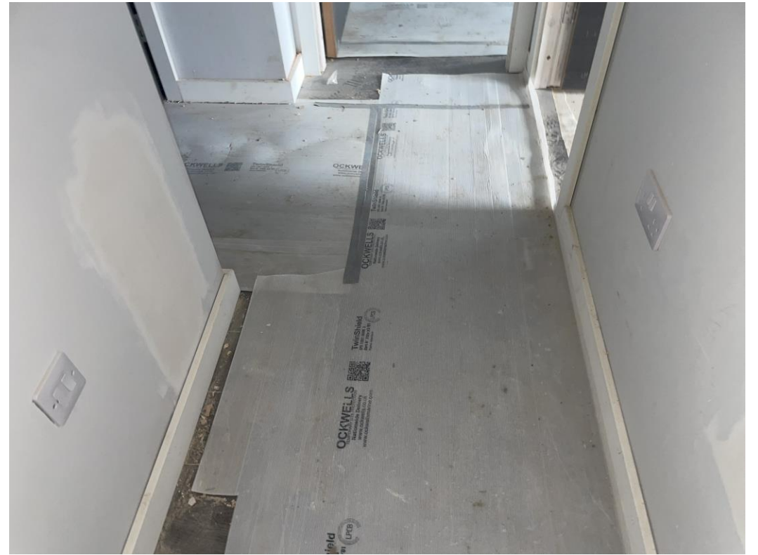
Level 2 – Laminate installed
