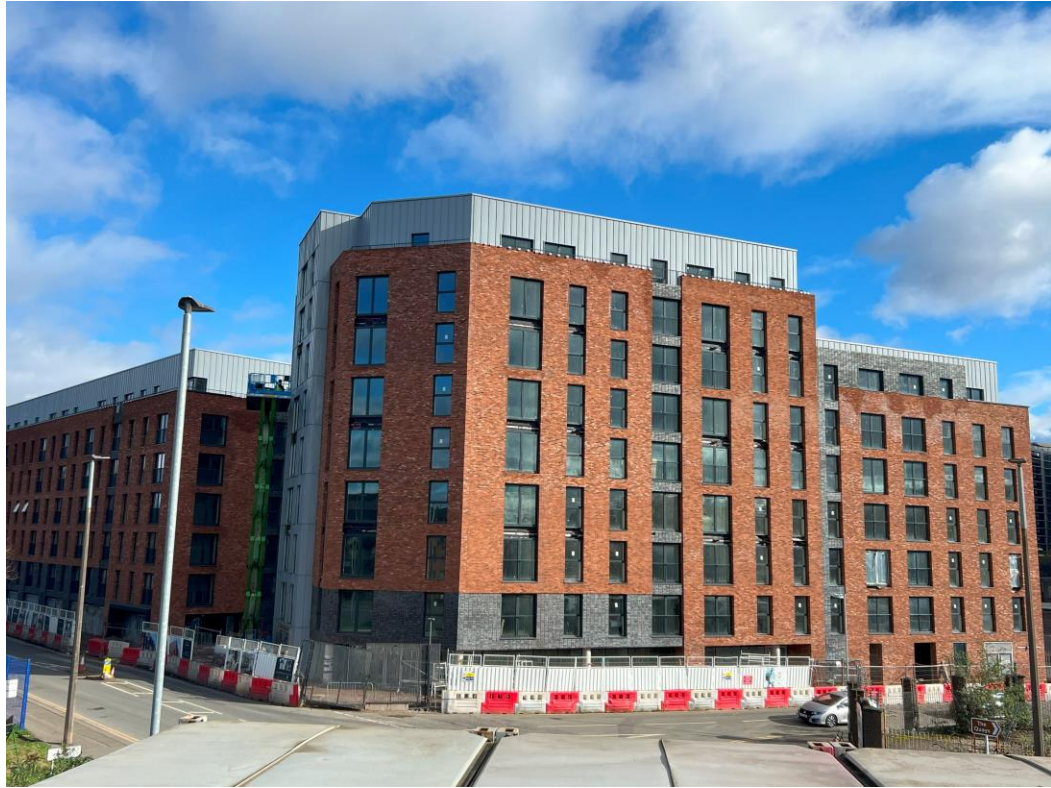
Ordsall Lane site view
