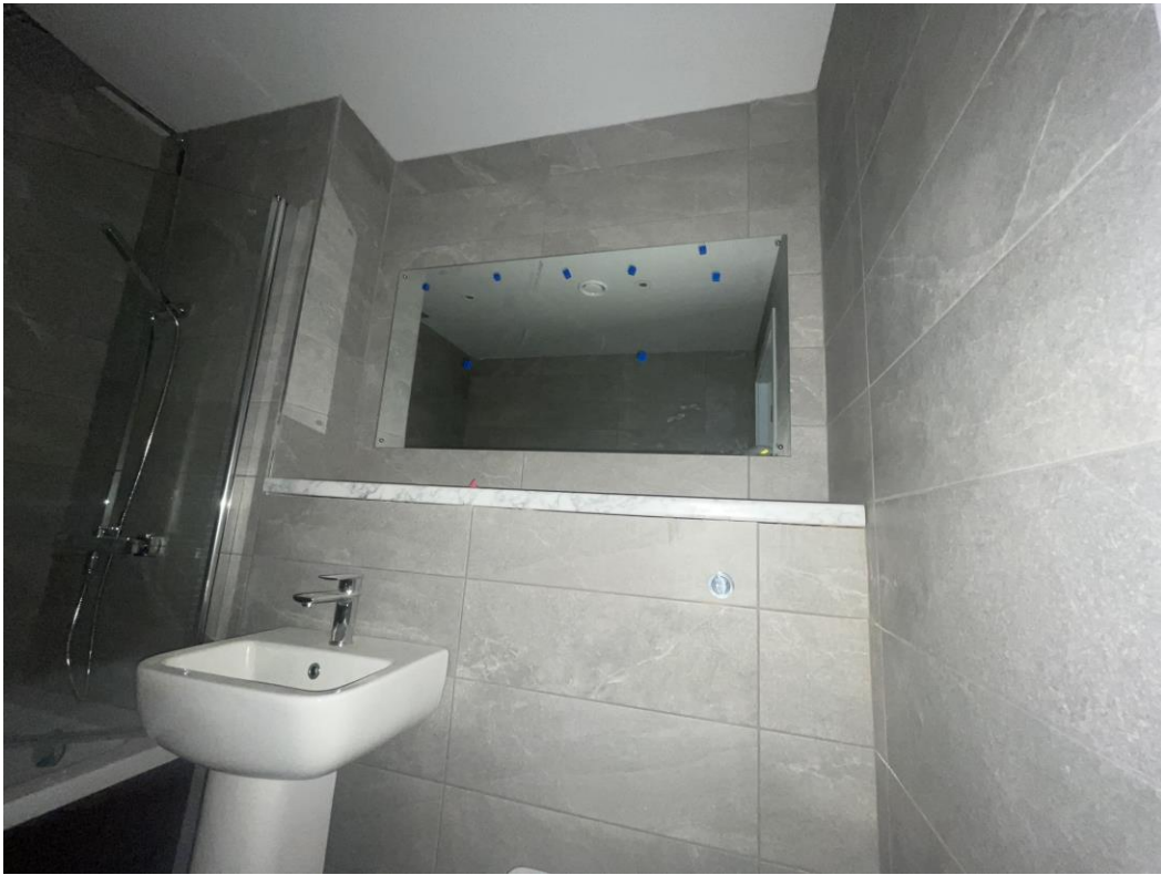
Level 6 – Mirror installed
