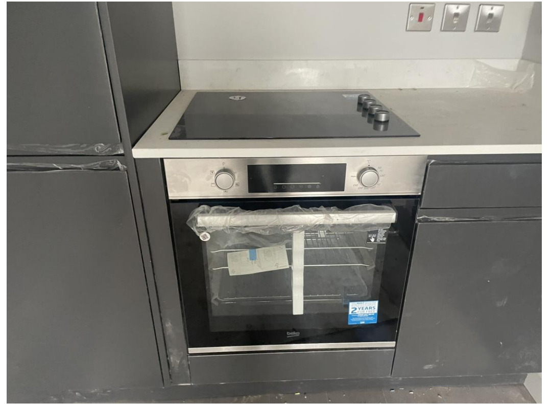
Level 8 – Appliances installed
