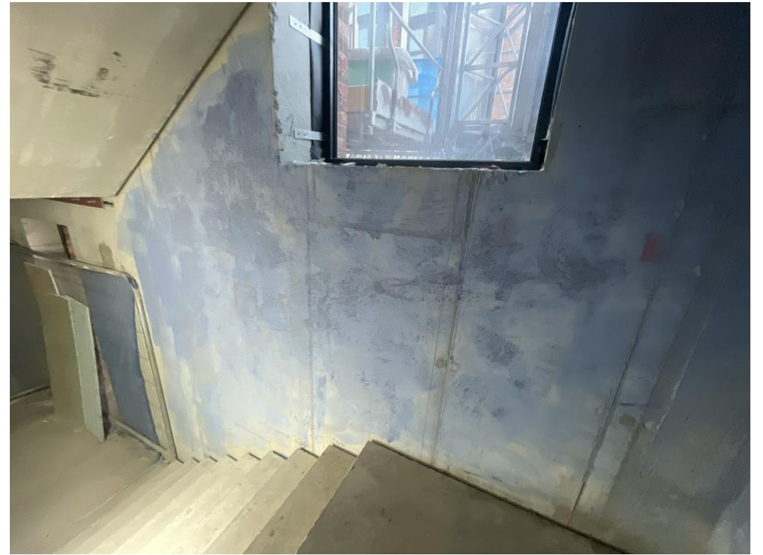
Block A – Blue grit adhesive applied to walls
