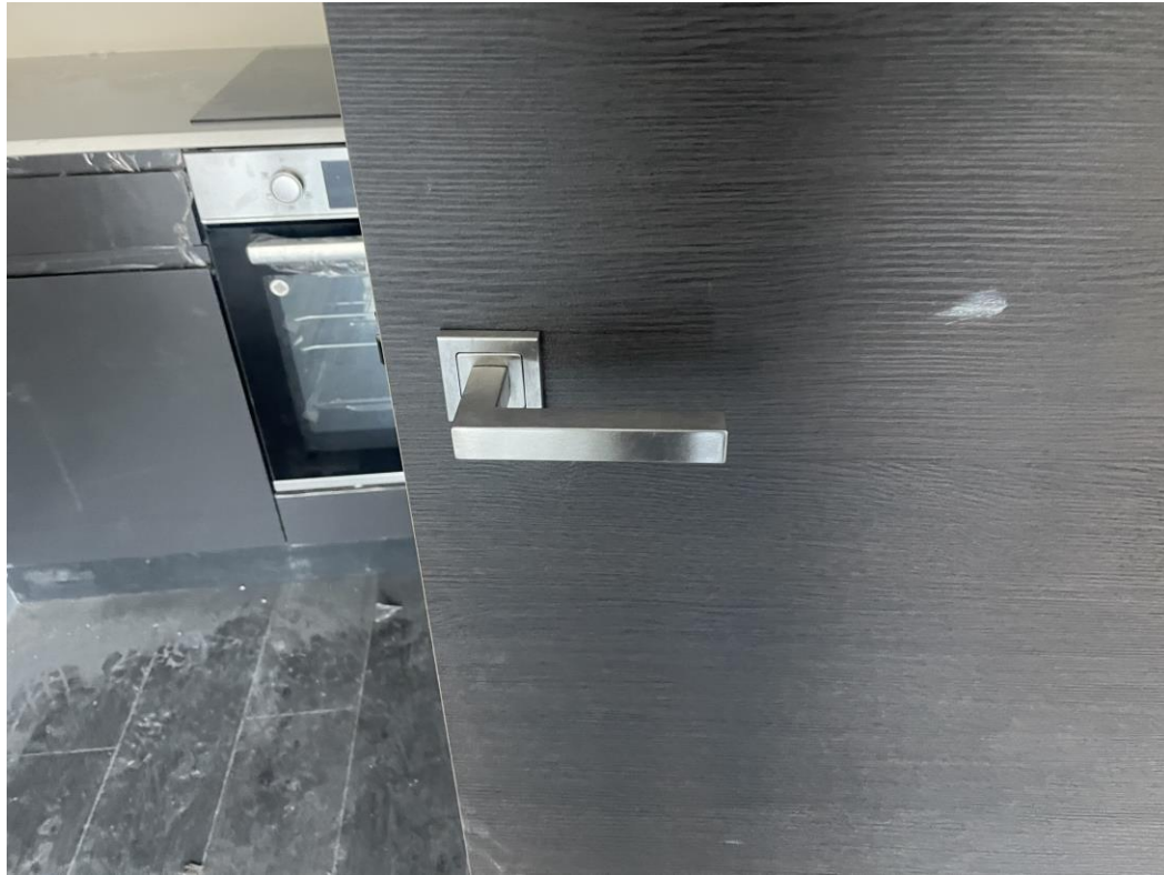
Level 1 – Ironmongery installed
