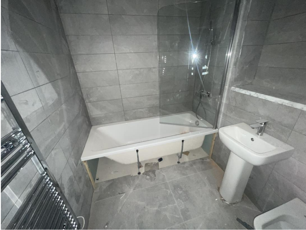
Level 5 – Sanitary items installed
