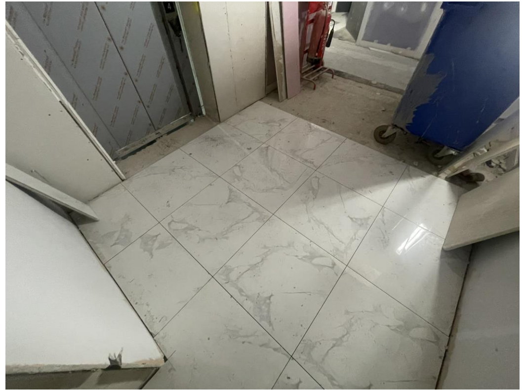
Level 4 - Lift lobby floor tiling
