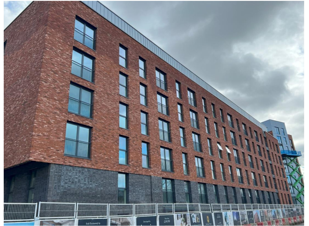
Ordsall Lane site view
