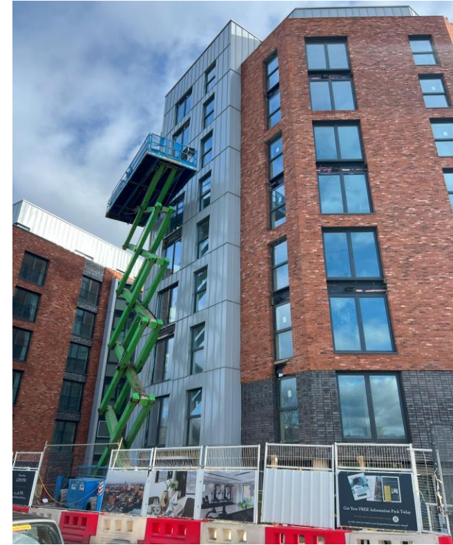
Ordsall Lane site view
