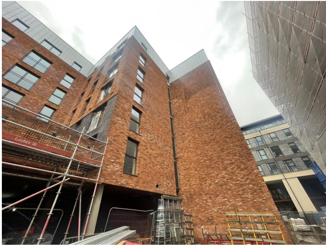
Podium site view
