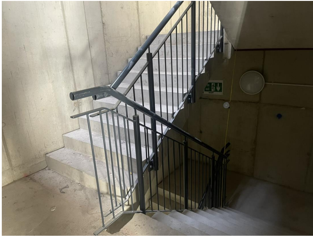
Level 4 - Stairwell balustrades
