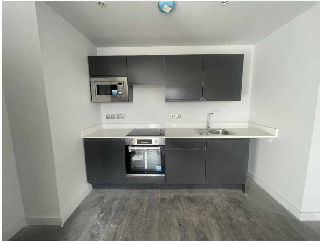
Level 6 – Kitchen units & worktop installed
