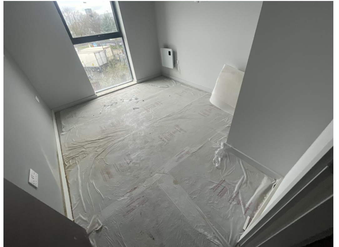
Level 5 – Carpet installed
