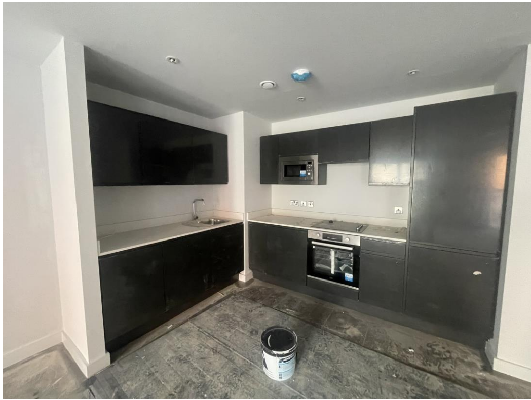
Level 1 – Kitchen units installed
