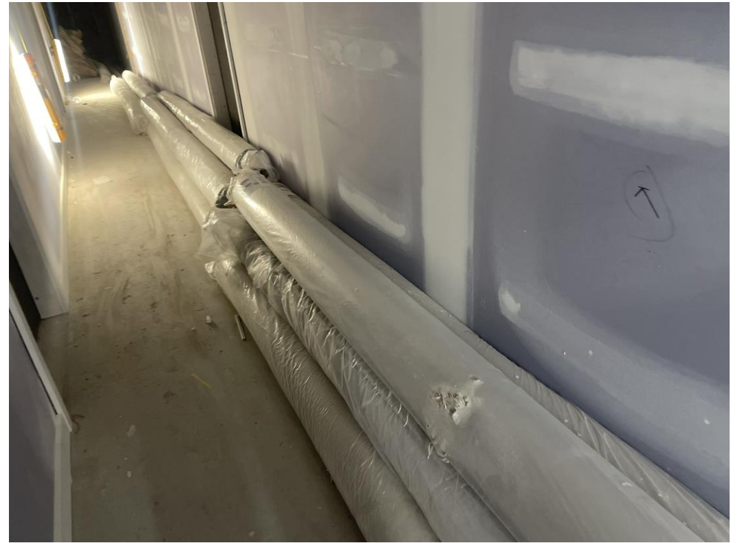
Level 3 – Carpets loaded for isallation
