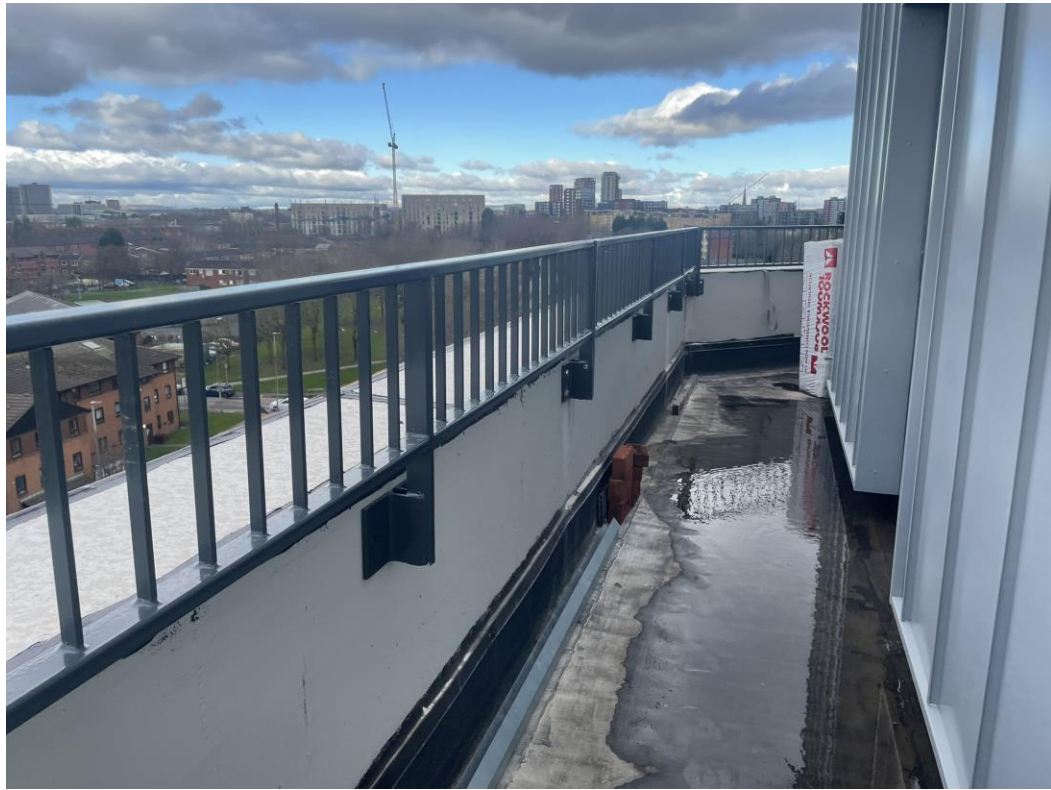
Block A Balustrade handrail
