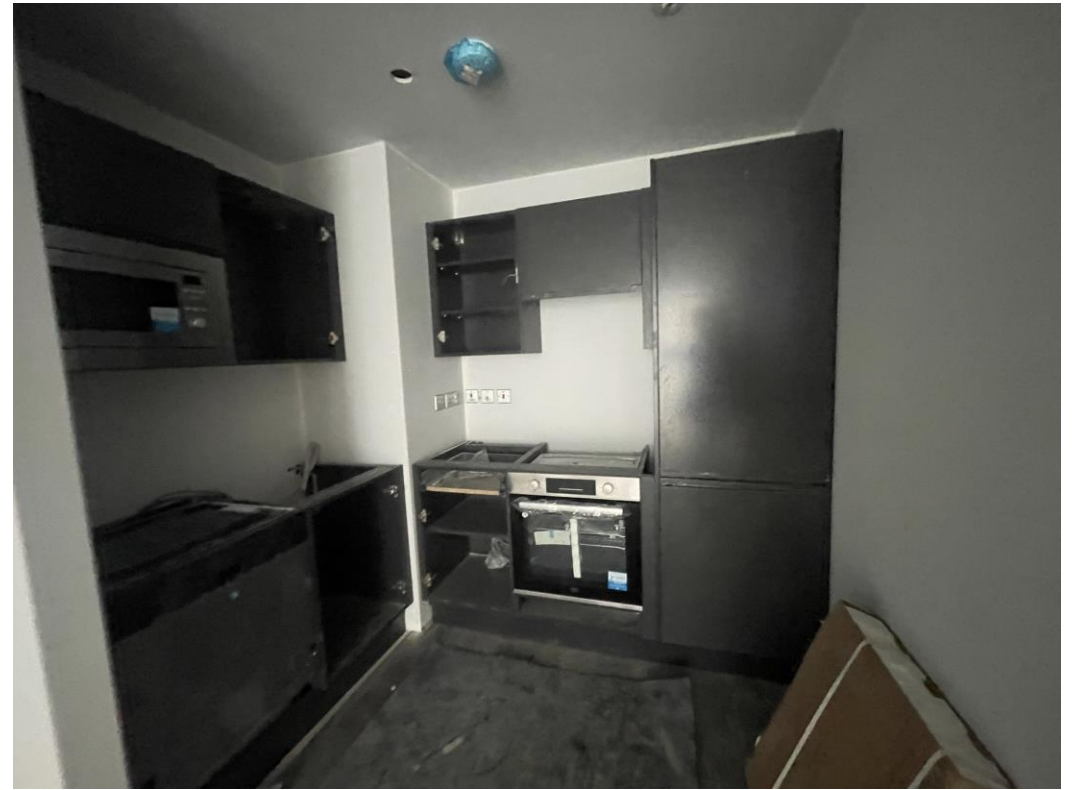
Level 6 – Kitchen units
