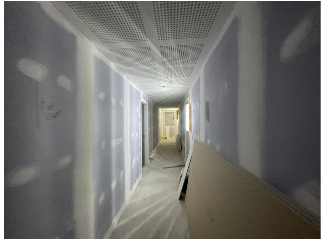
Level 4 – Acoustic ceiling decoration corridor
