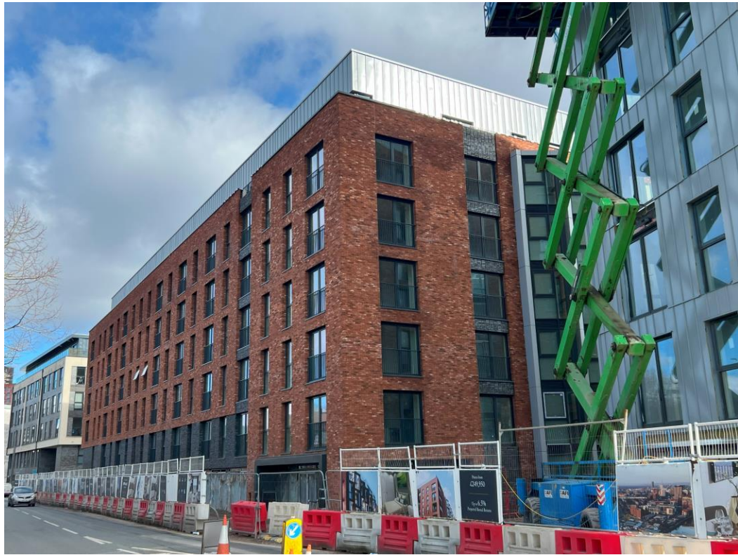
Ordsall Lane site view
