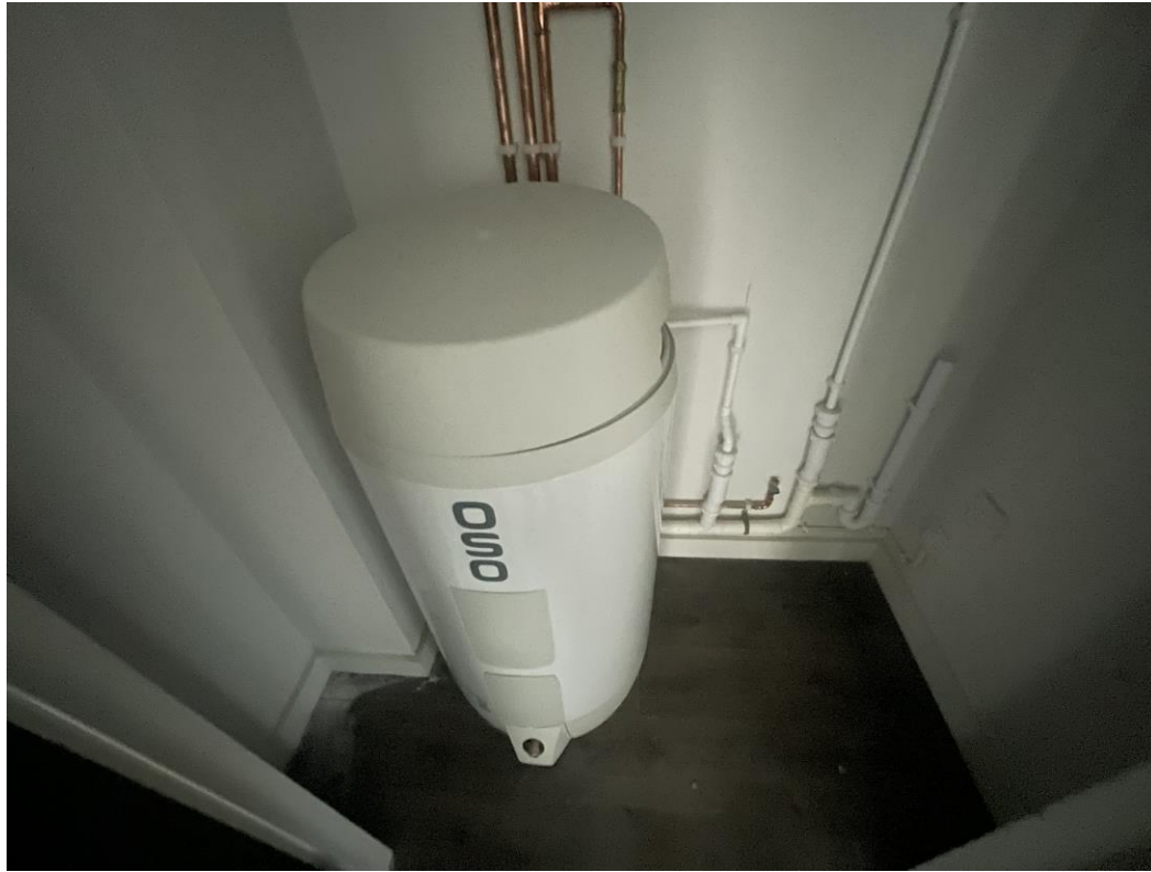
Level 3 – 2 nd fix mechanical & electrical
