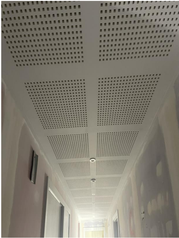
Level 3 – Acoustic ceiling decoration corridor
