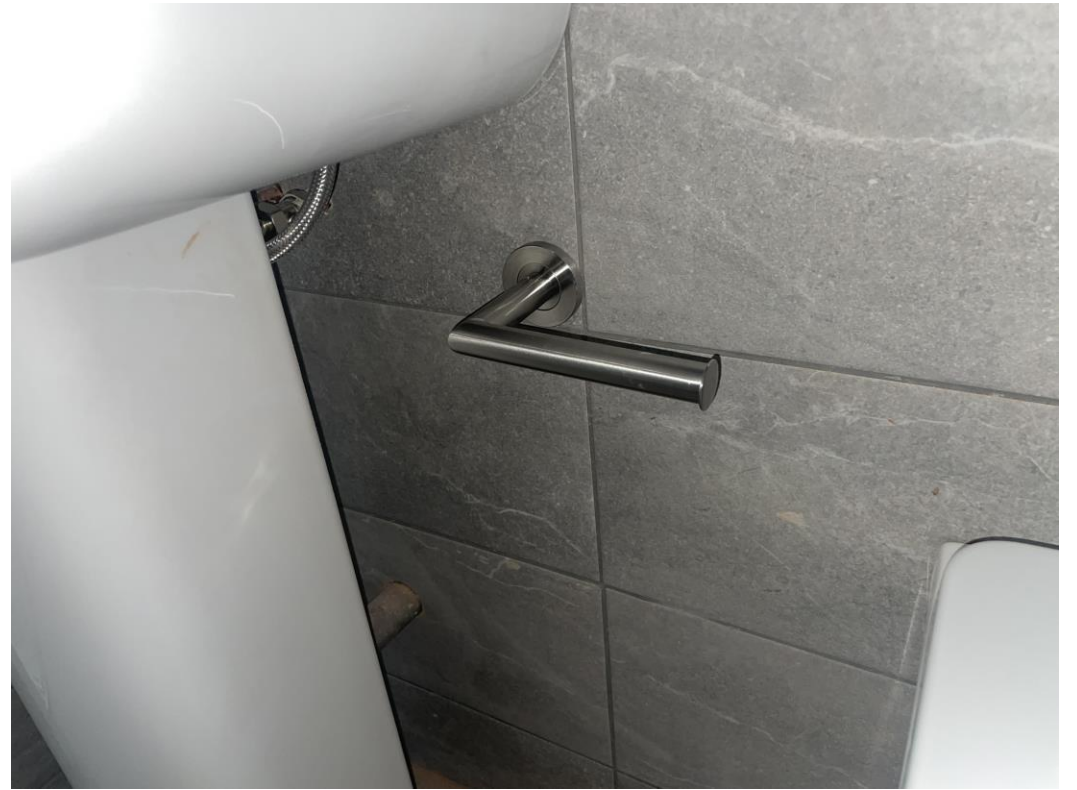
Level 6 – Fittings installed
