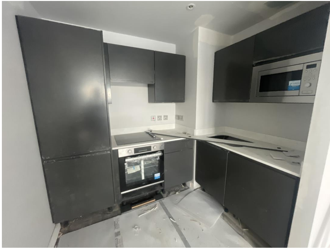
Level 5 – Kitchen complete
