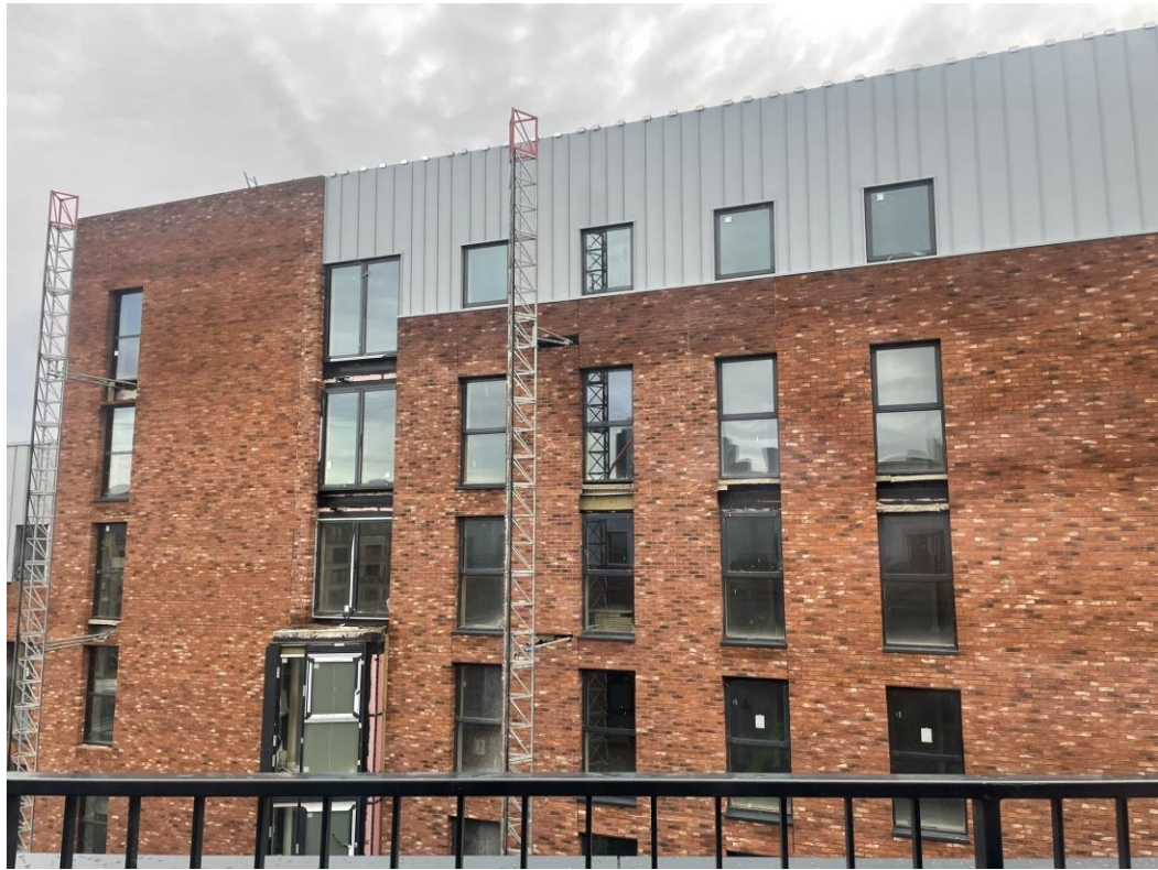
Block B wall insulation and cladding
