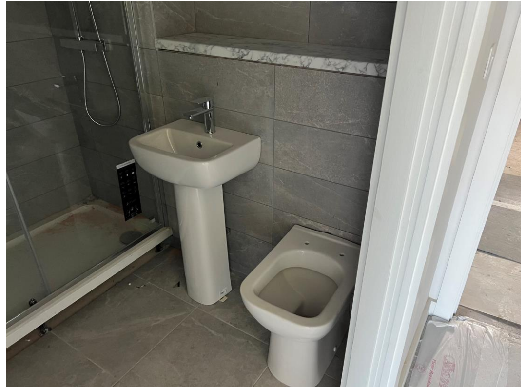
Level 5 – vanity top installed
