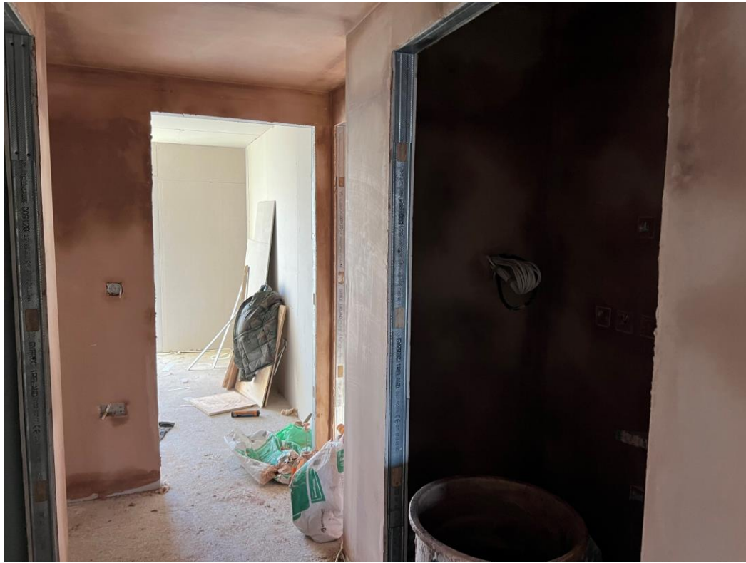
Level 6 – Hoist apartment plaster skim finish
