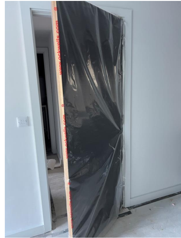
Level 2 – Apartment doors installed
