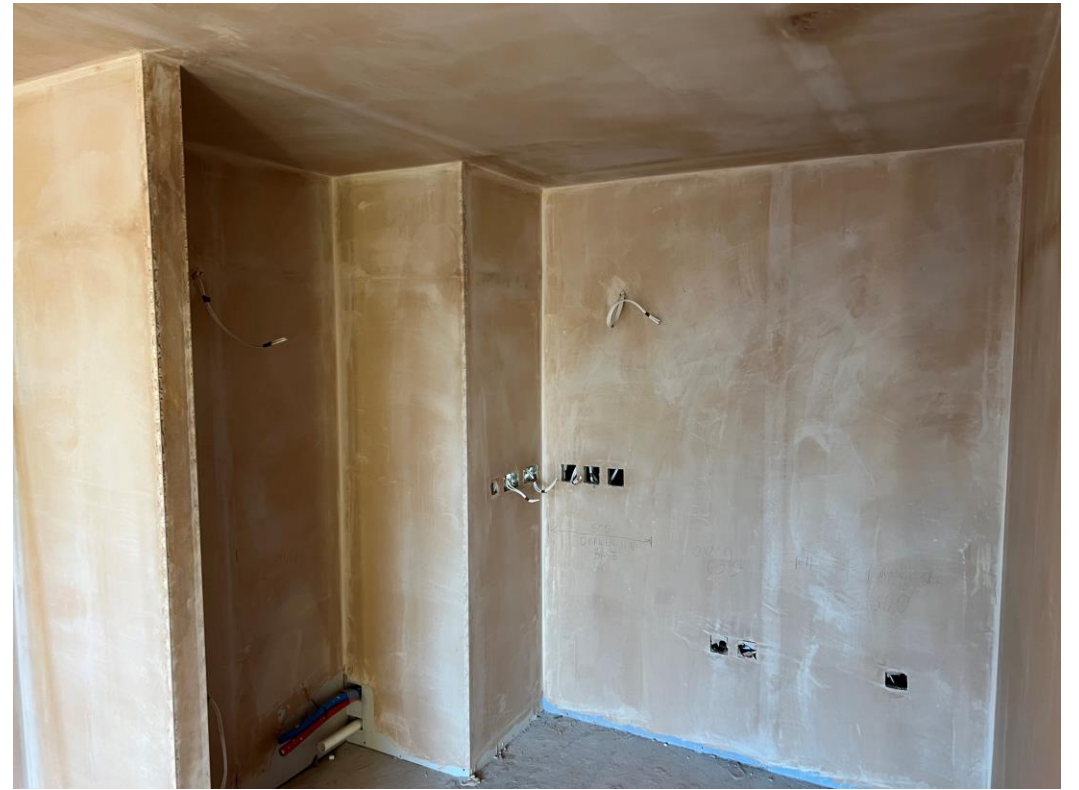
Level 8 – Hoist apartment plaster skim finish
