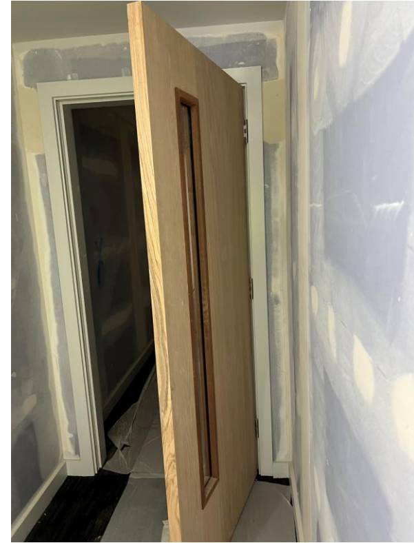
Level 6 – corridor door installed
