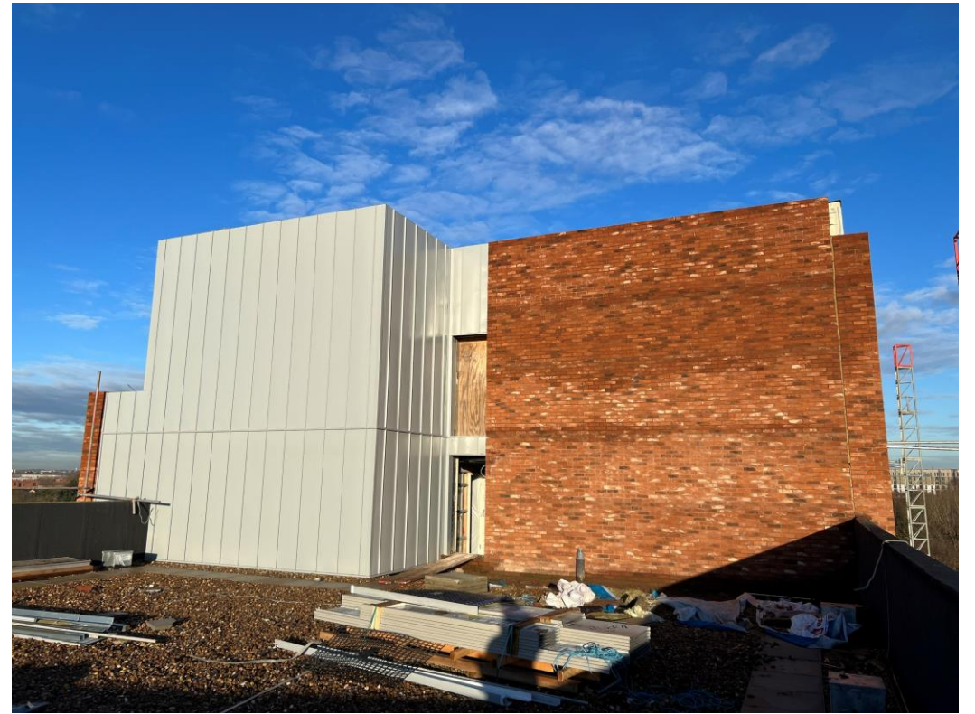
Block A wall insulation and cladding
