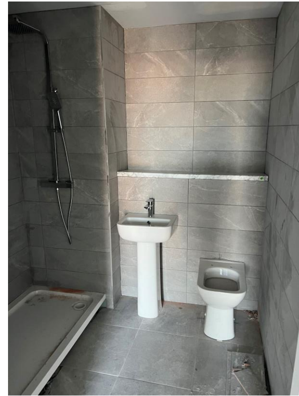
Level 4 – vanity top installed
