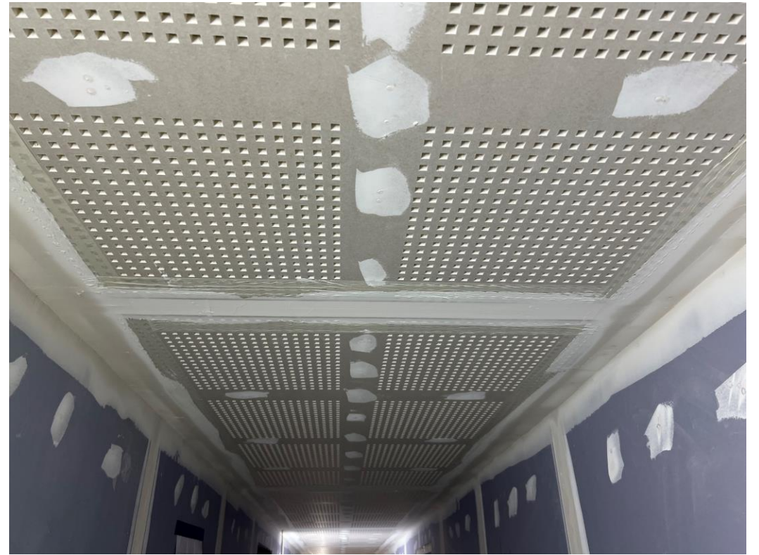
Level 4 – acoustic ceiling decoration corridor
