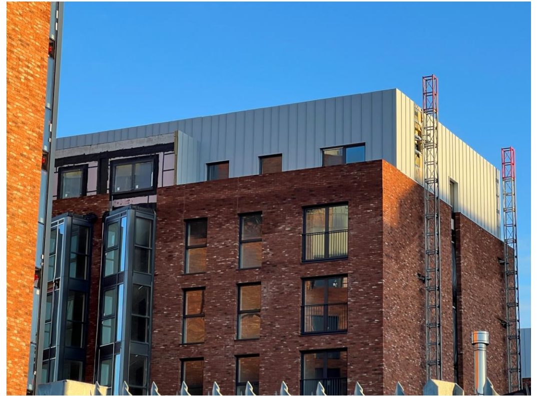
Worrall Street site view
