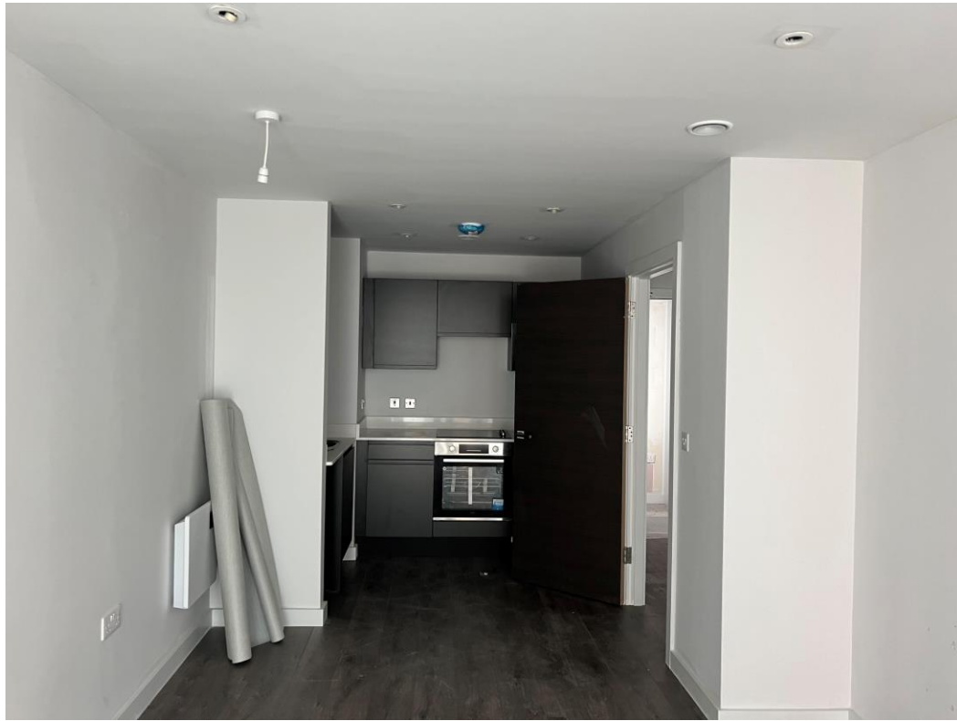
Level 4 – Kitchen units installed
