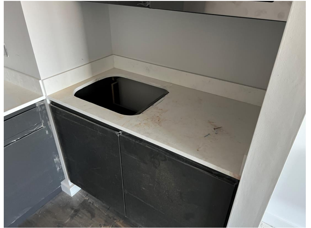
Level 6 – Kitchen units & worktops installed
