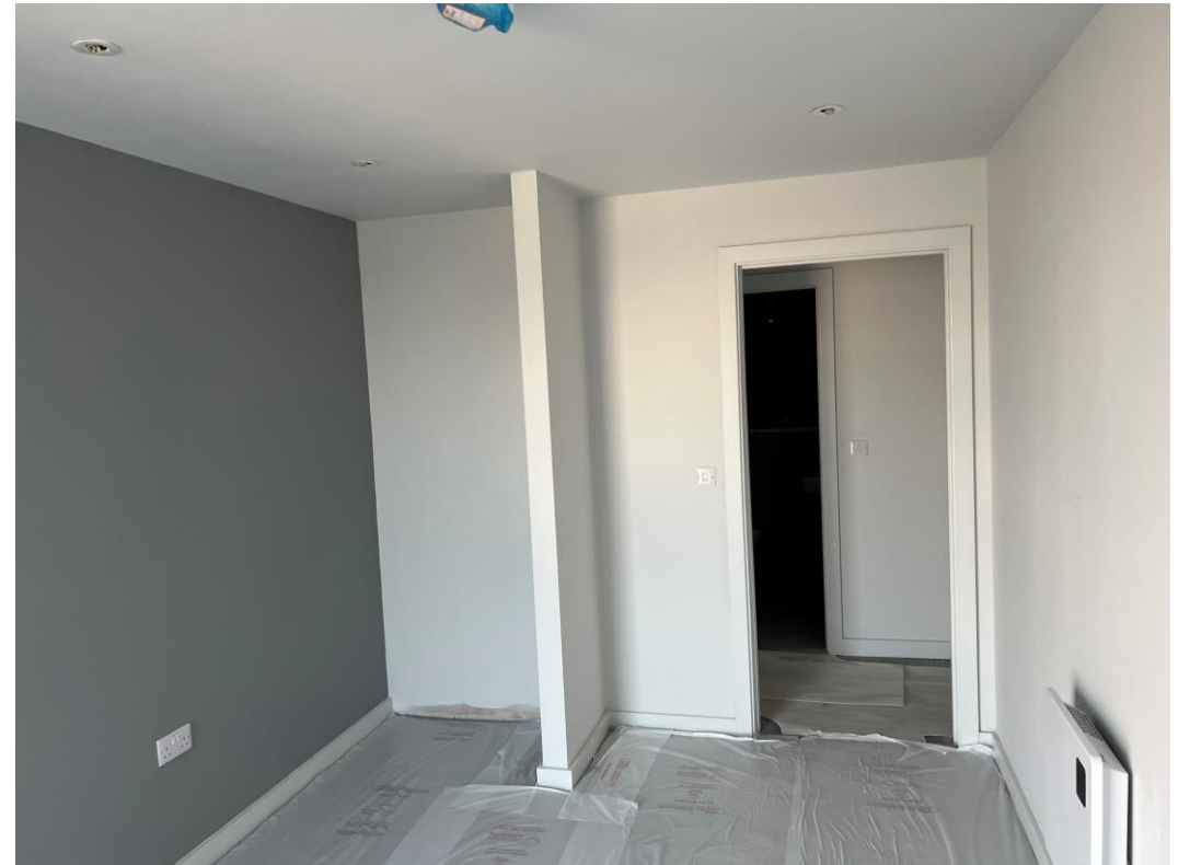
Level 5 – feature wall finish
