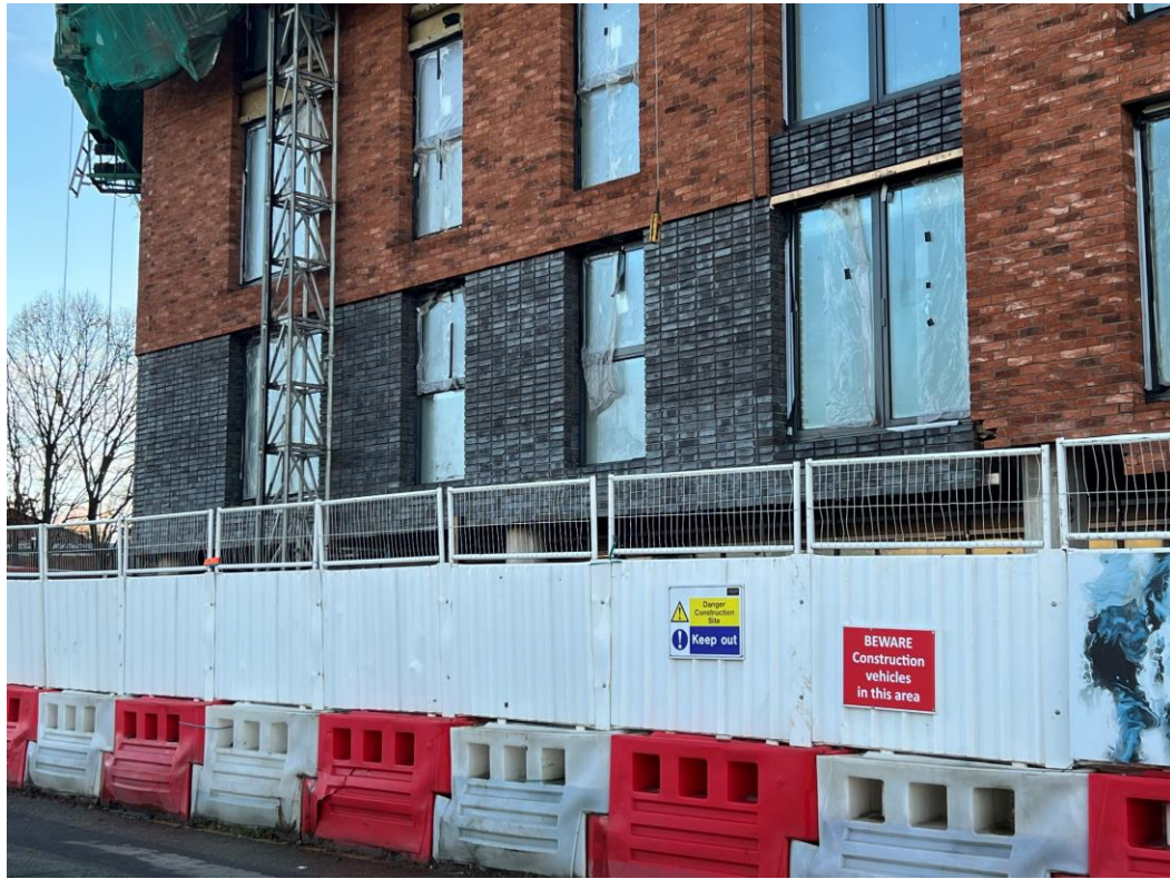
Worrall Street site view
