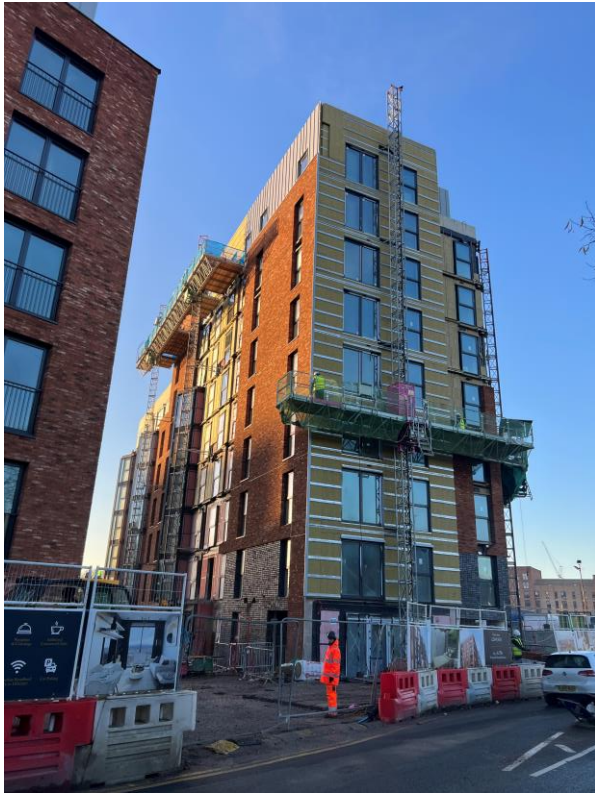
Ordsall Lane site view
