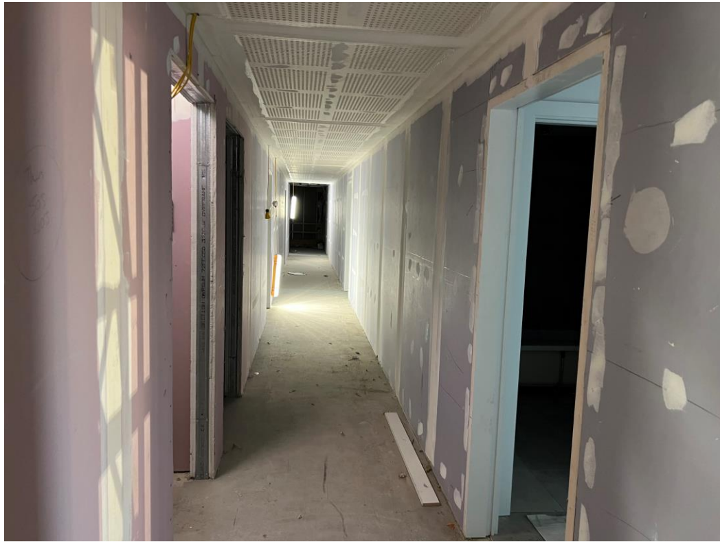
Level 4 – acoustic ceiling decoration corridor
