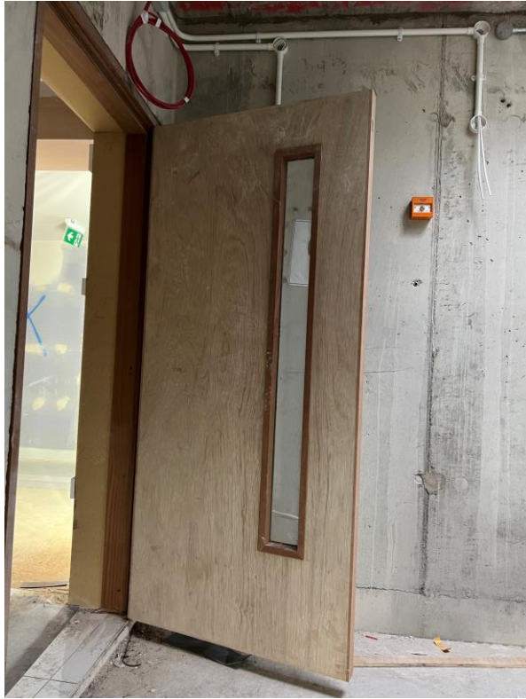
Level 6 – door to stairwell
