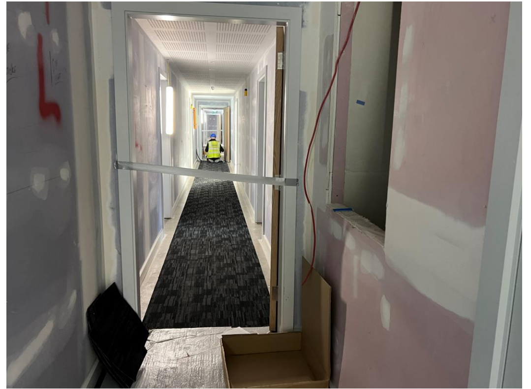
Level 3 – corridor carpet
