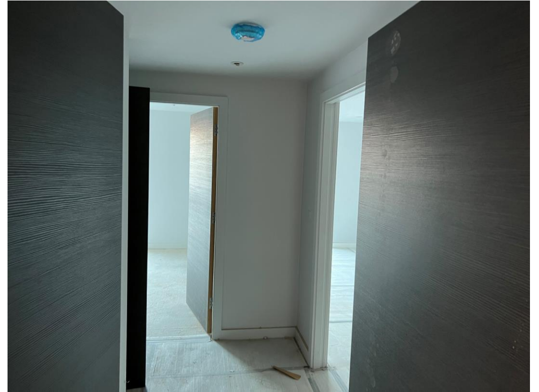
Level 1 – Apartment doors installed
