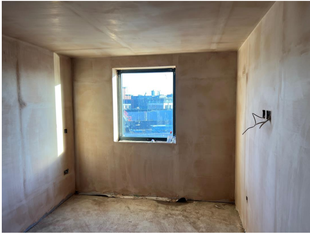
Level 8 – Hoist apartment plaster skim finish
