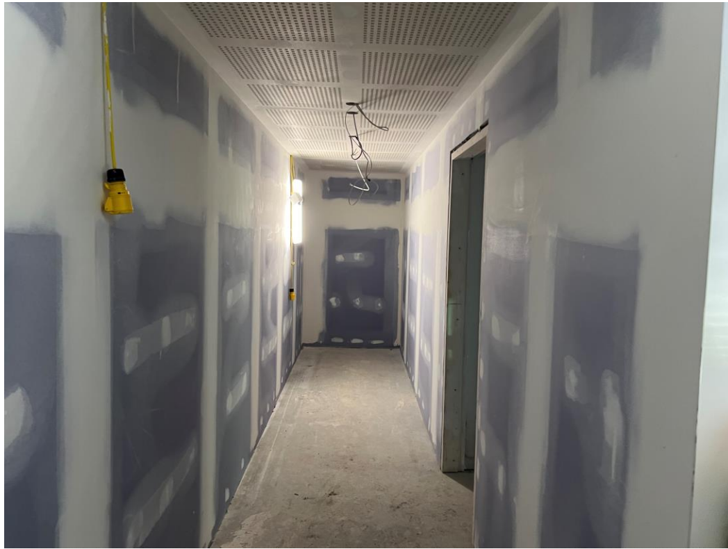
Level 1 – corridors boarded ready for decoration
