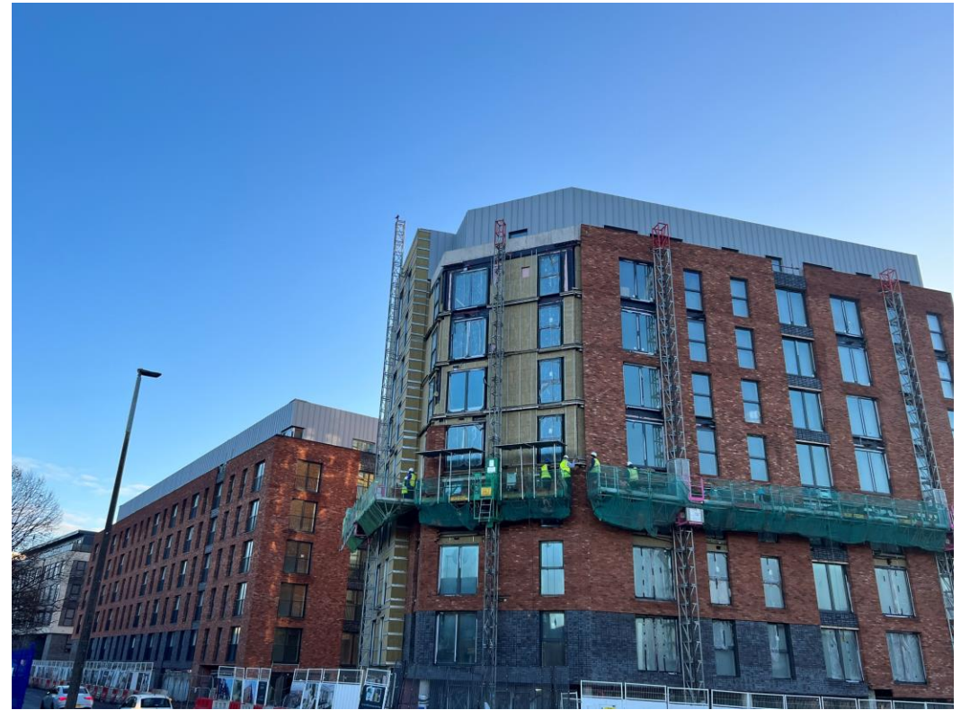
Ordsall Lane site view
