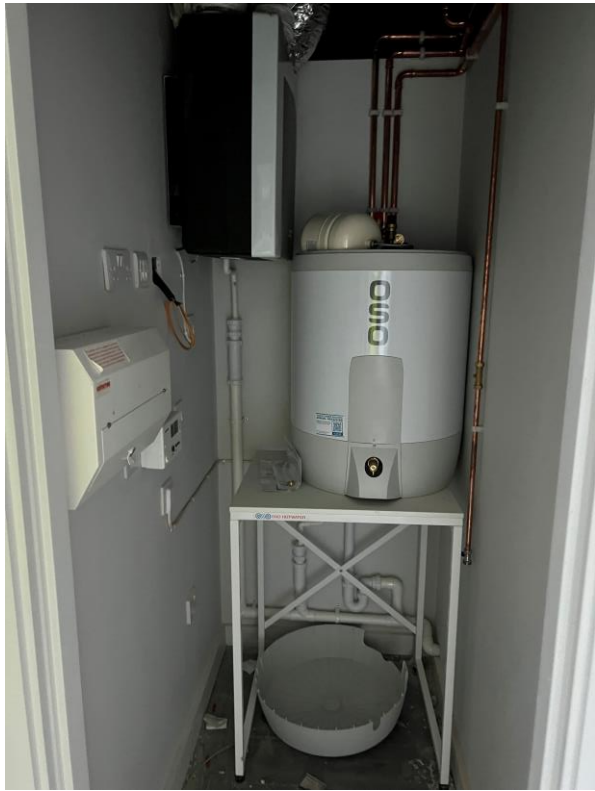
Level 3 – 2 nd fix mechanical & electrical
