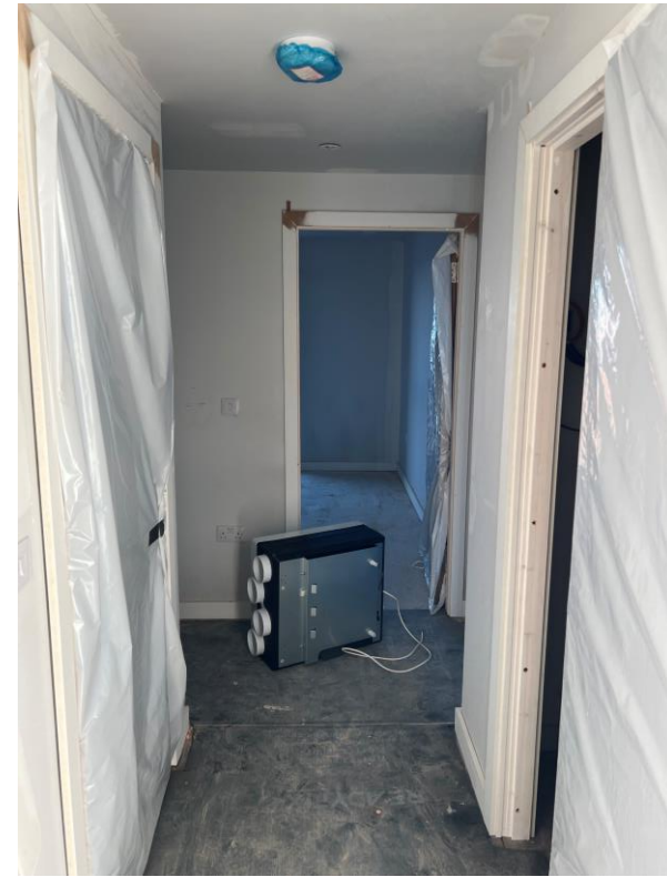
Level 7 – Internal doors installed
