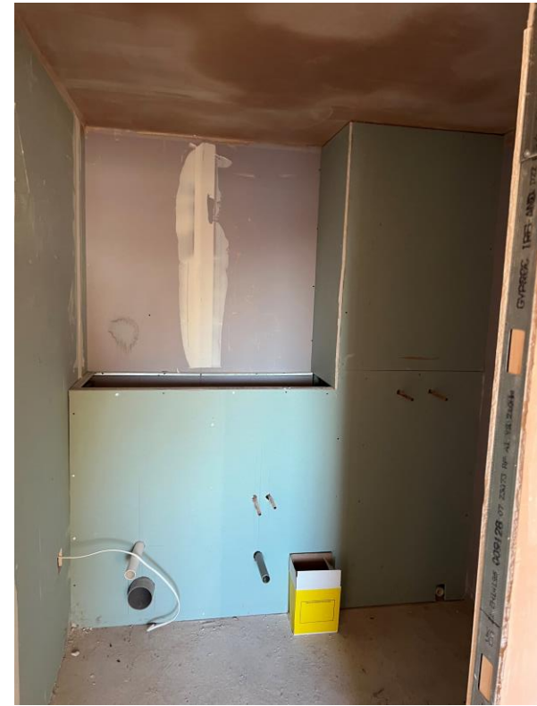
Level 8 – Hoist apartment plaster skim finish
