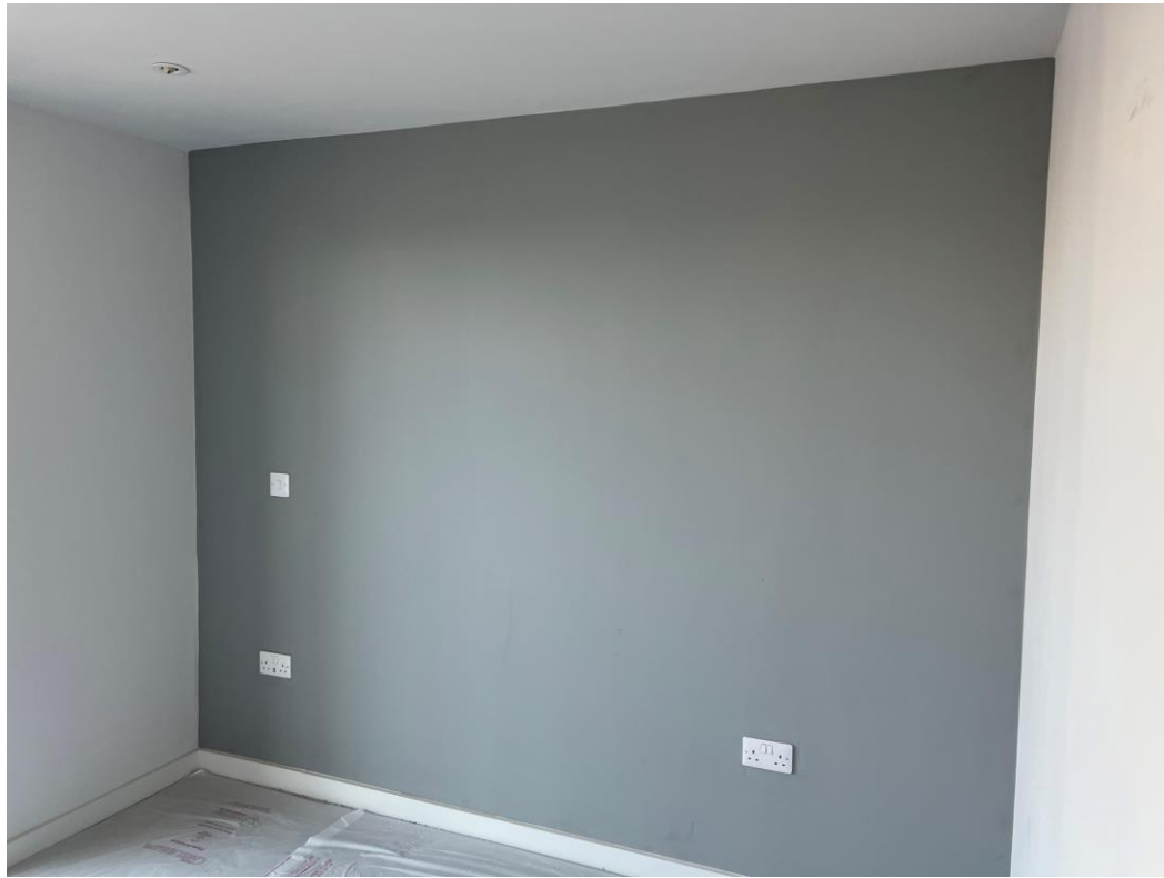
Level 5 – feature wall finish
