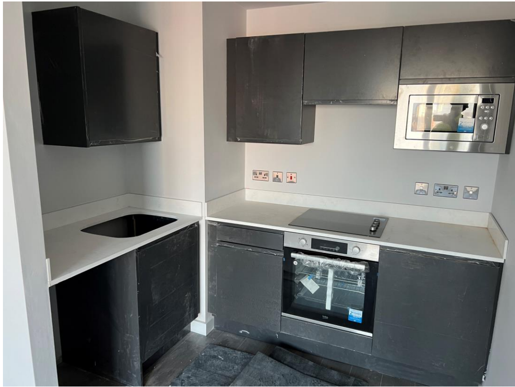
Level 6 – Kitchen units & worktops installed
