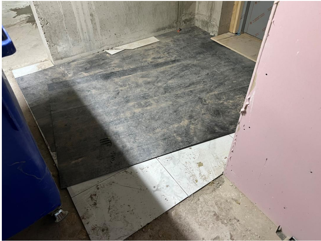
Level 3 – floor tiling lift lobby
