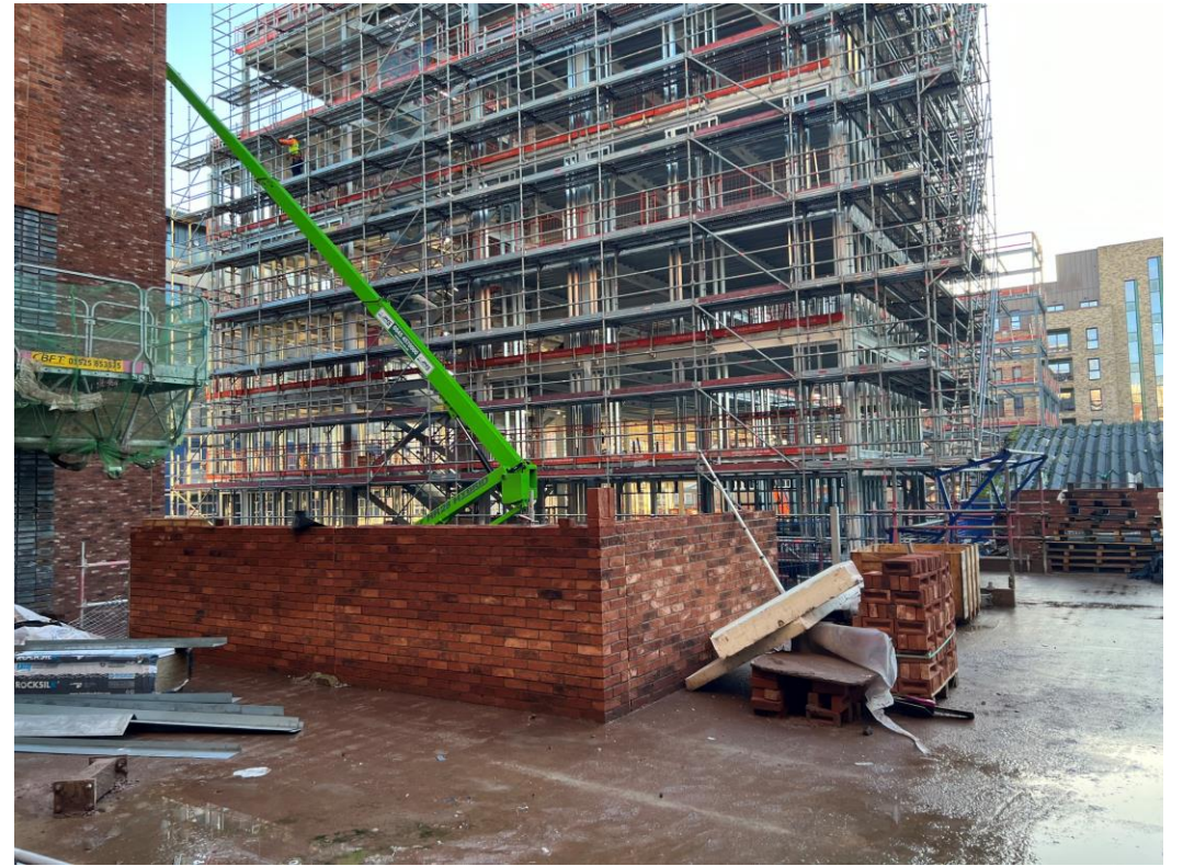
Block B brickwork parapet
