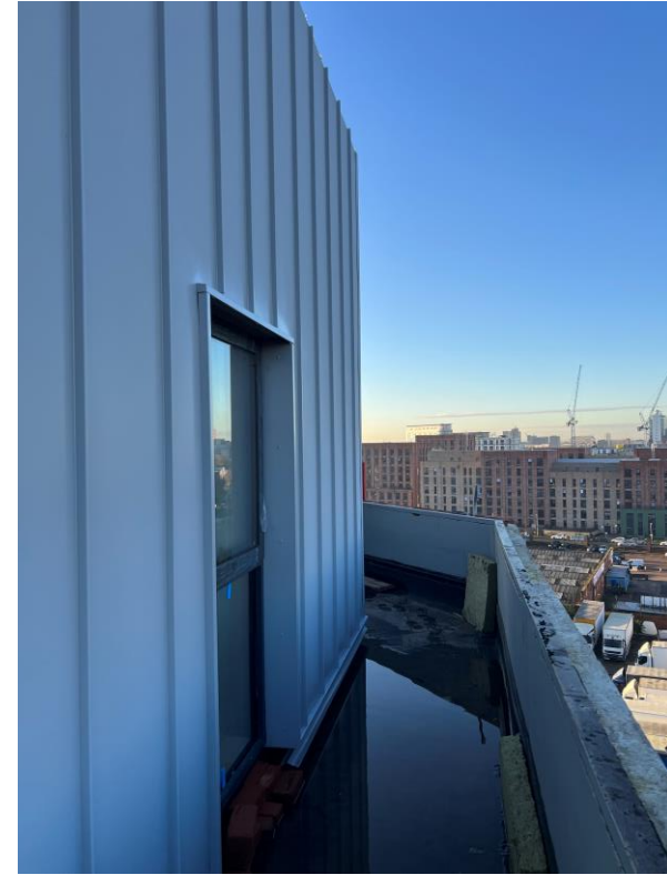
Block A wall cladding
