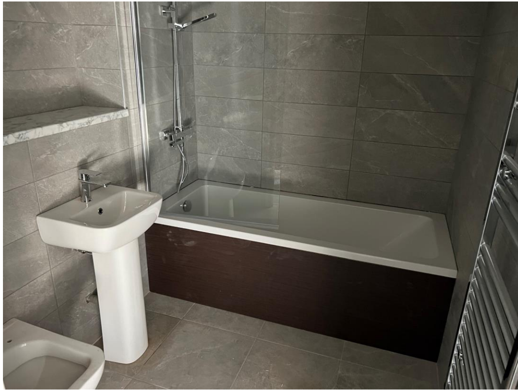
Level 6 – Sanitary appliances installed
