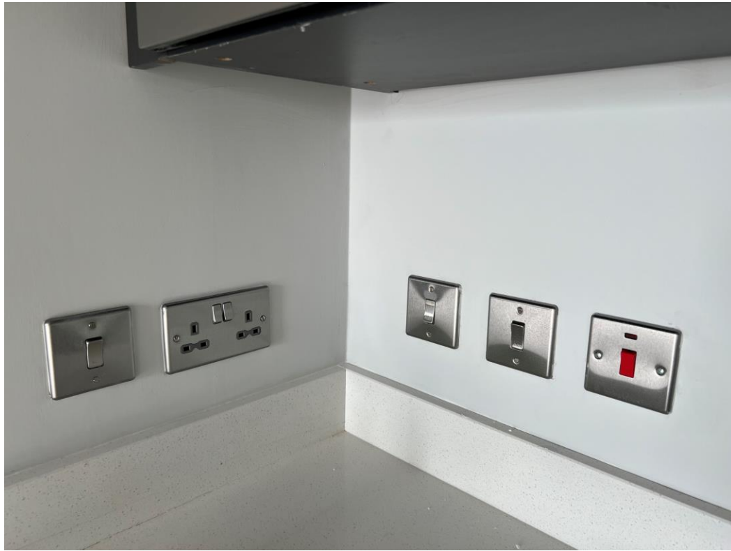
Level 6 – Second fix electrical
