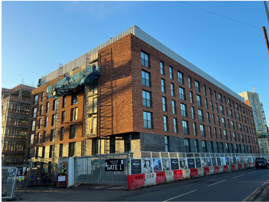
Ordsall Lane site view
