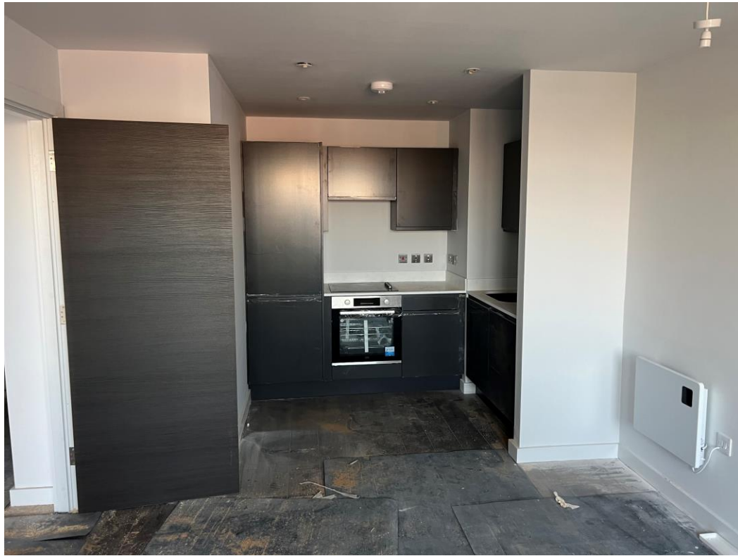
Level 6 – Internal doors installed
