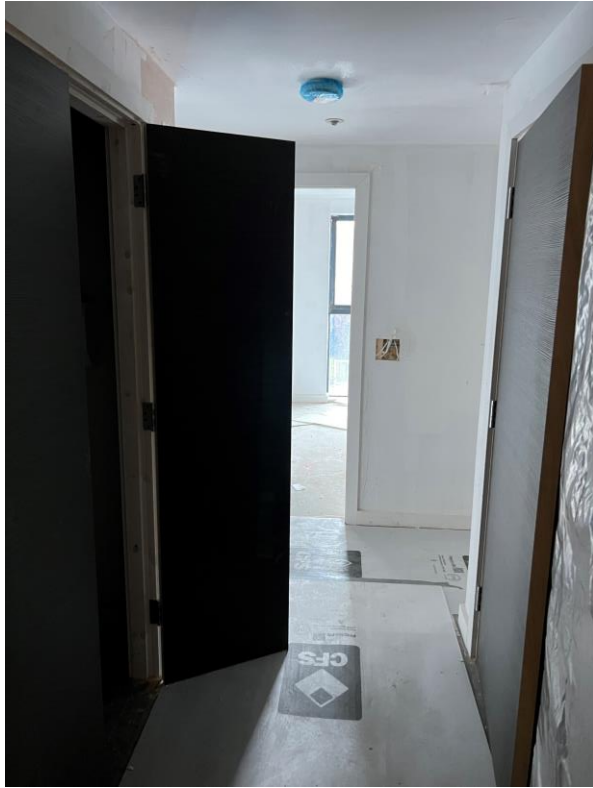
Level 1 – Apartment doors installed
