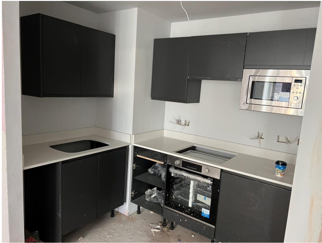
Ground Level – Kitchen units installed
