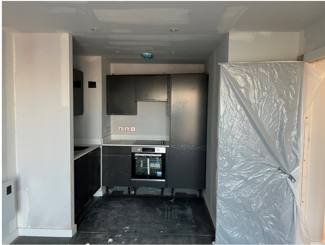
Level 7 – Internal doors installed
