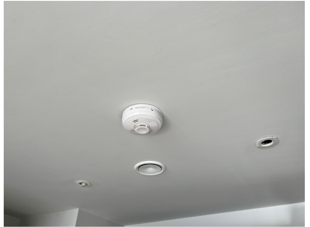
Level 6 – Second fix electrical
