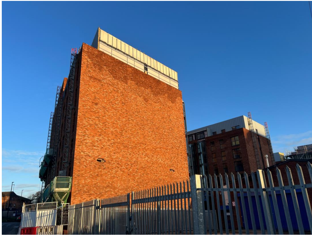
Worrall Street site view
