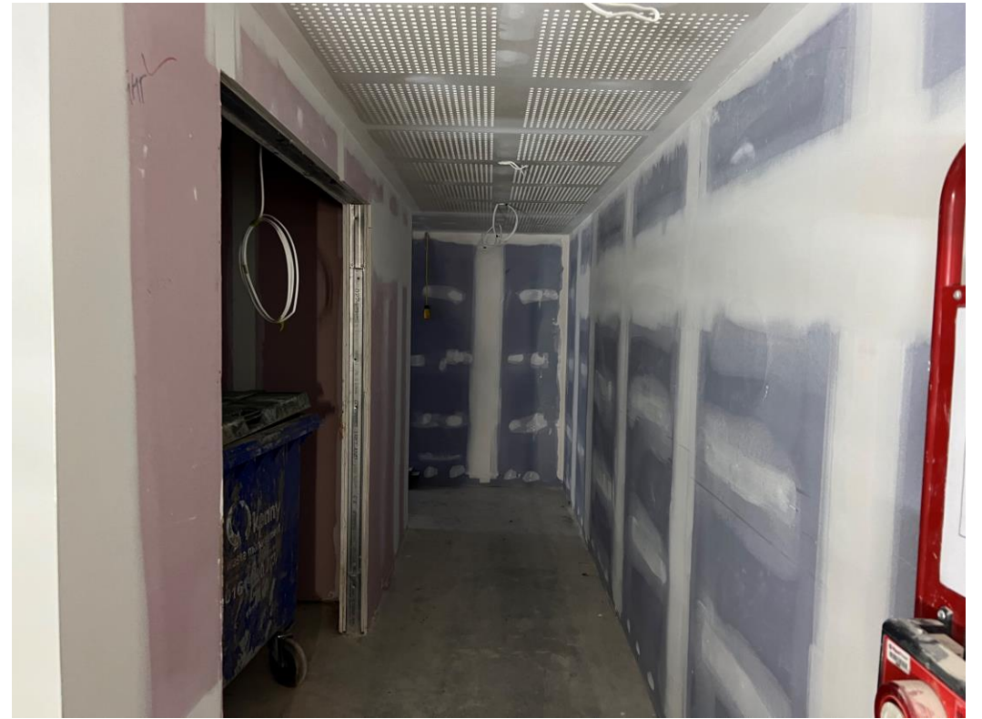
Level 1 – corridors boarded ready for decoration
