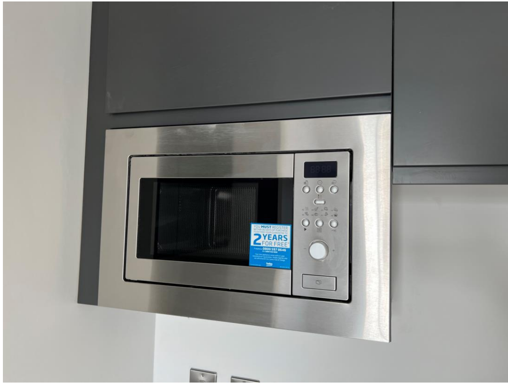
Level 6 – Kitchen appliances installed
