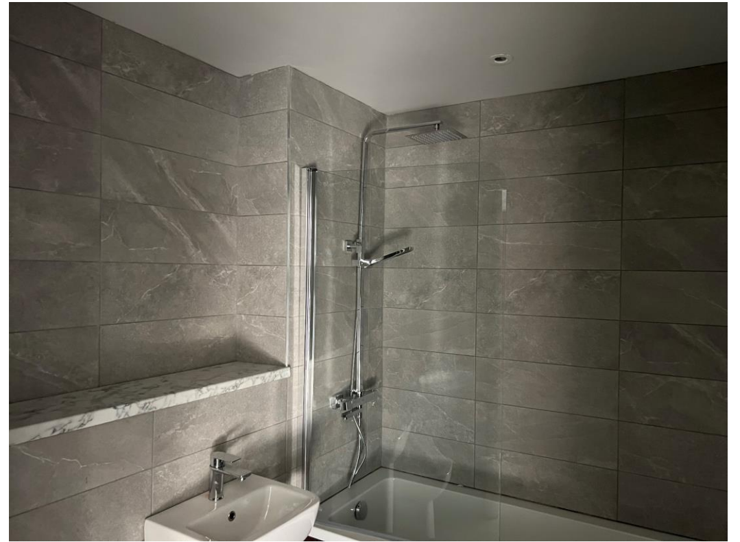
Level 6 – Sanitary appliances installed
