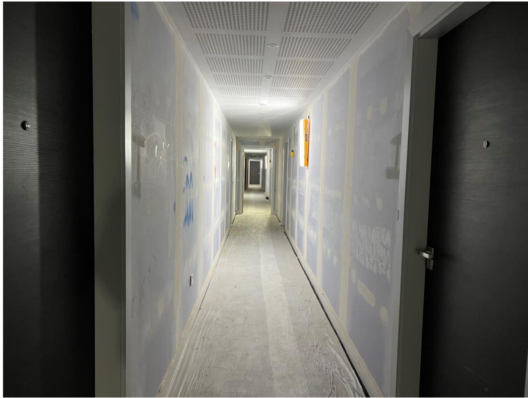
Level 5 – Apartment entrance door installed
