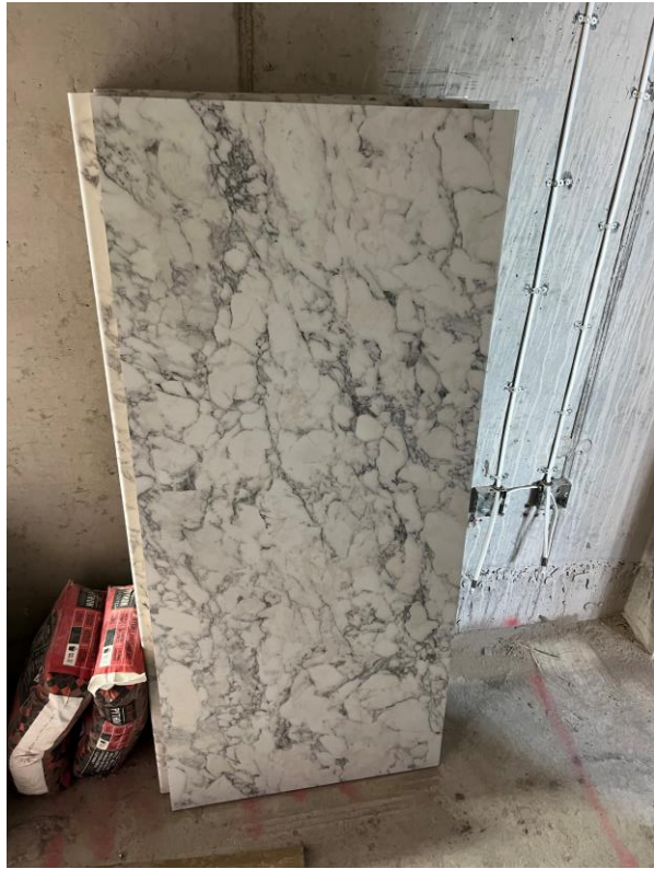
Level 5 – vanity top installed
