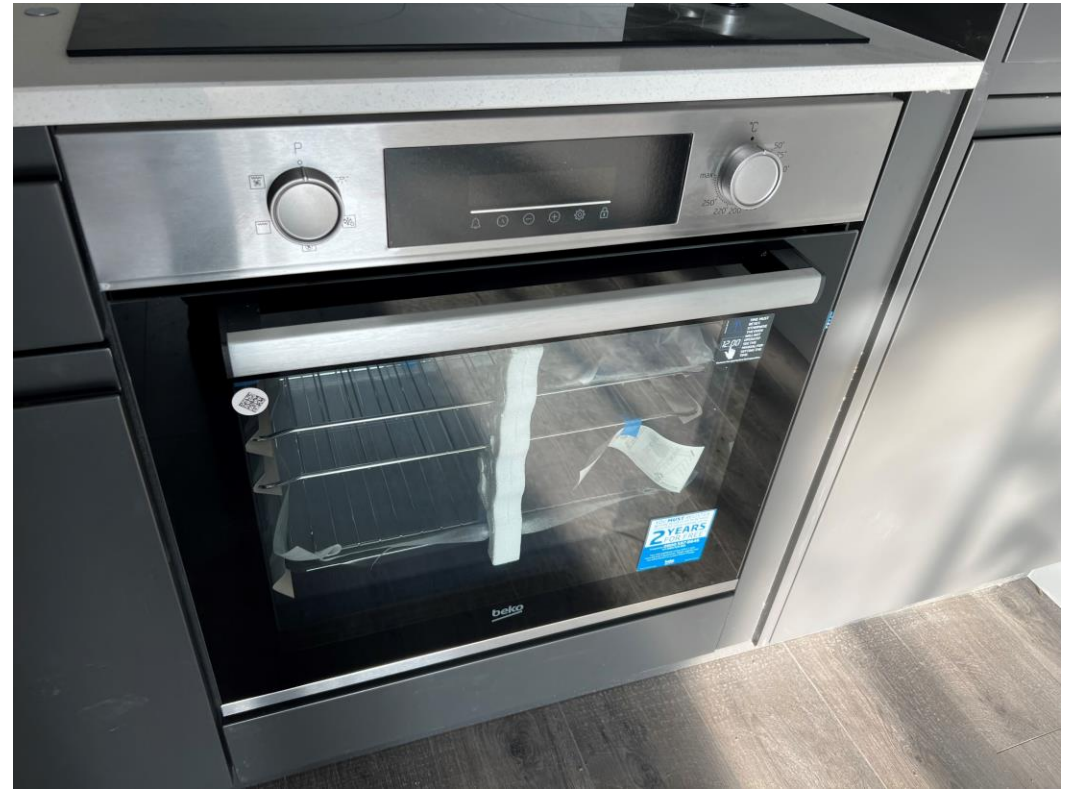
Level 6 – Kitchen appliances installed
