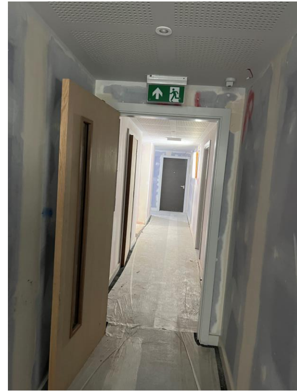
Level 6 – Apartment entrance door installed
