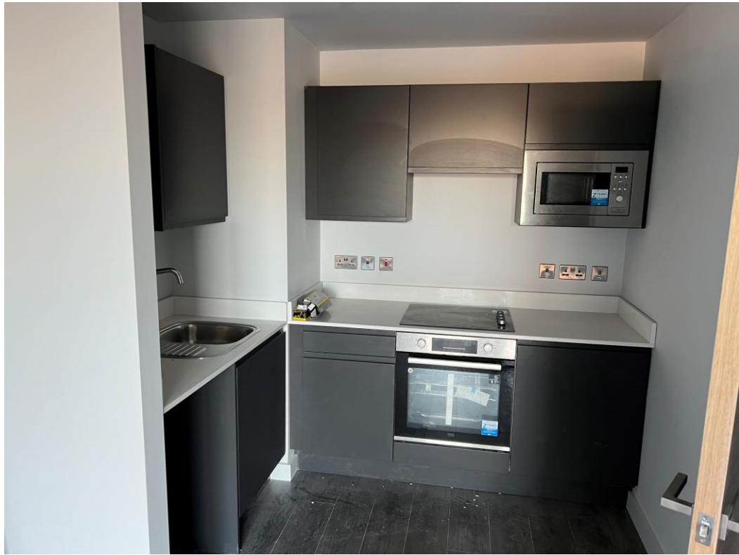
Level 5 – Kitchen units installed
