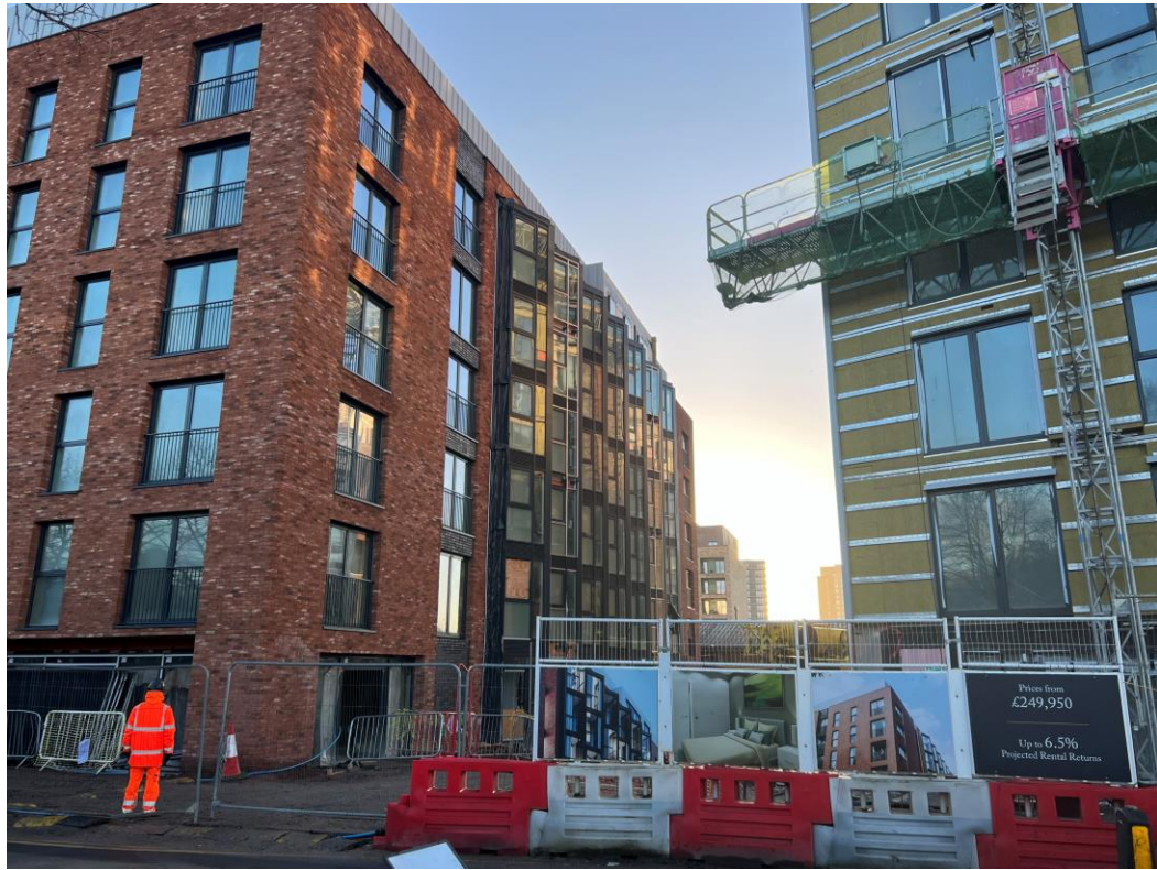
Ordsall Lane site view
