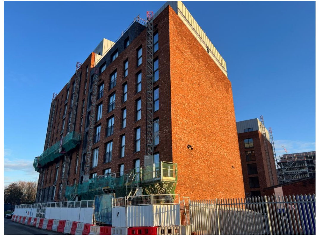
Worrall Street site view
