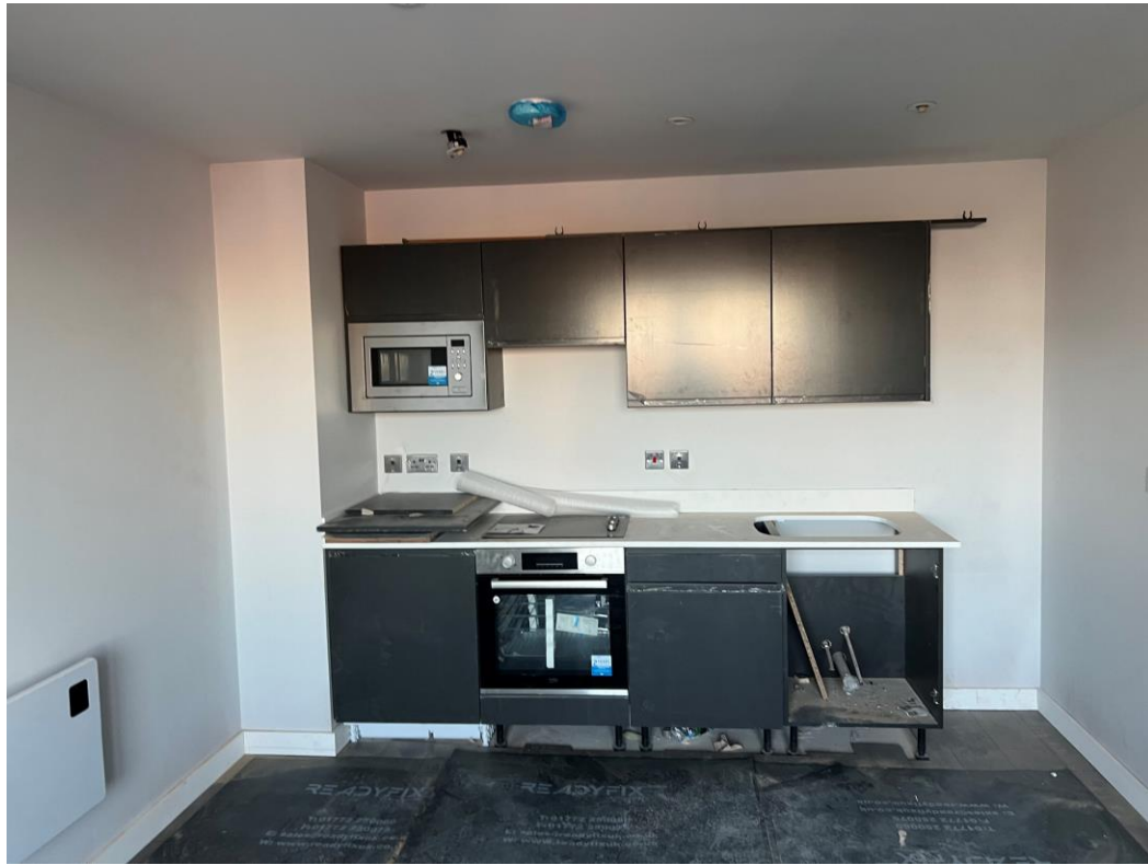
Level 8 – Kitchen units & worktops installed
