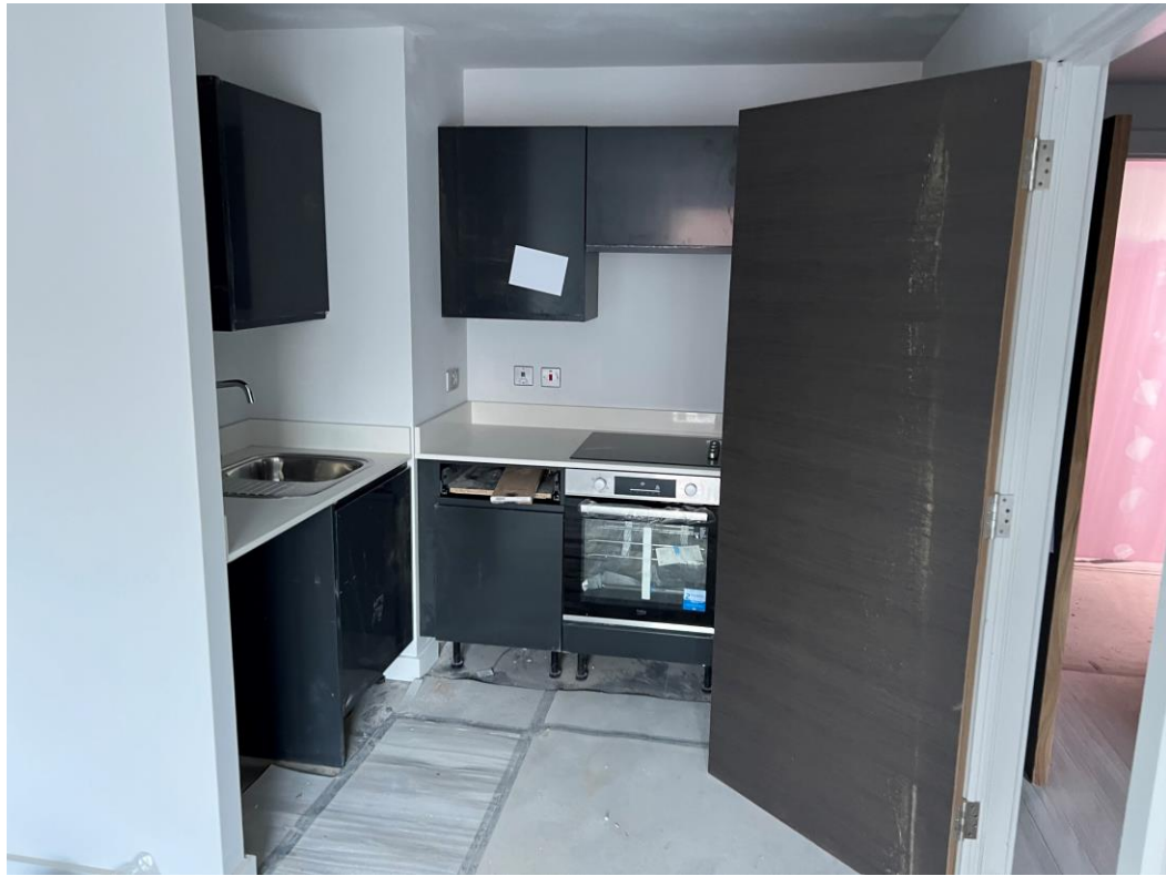
Level 2 – Kitchen units installed
