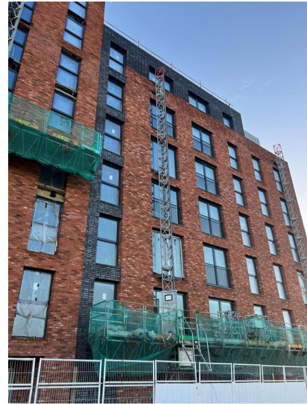
Worrall Street site view
