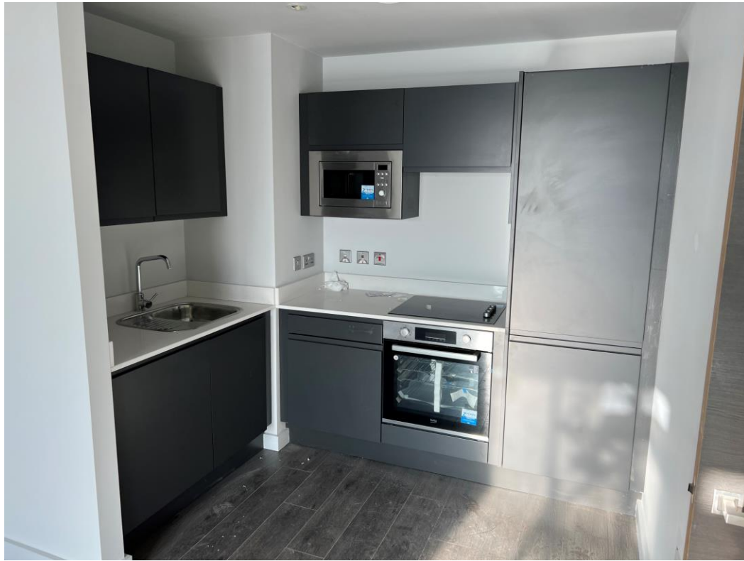
Level 6 – Kitchen units installed
