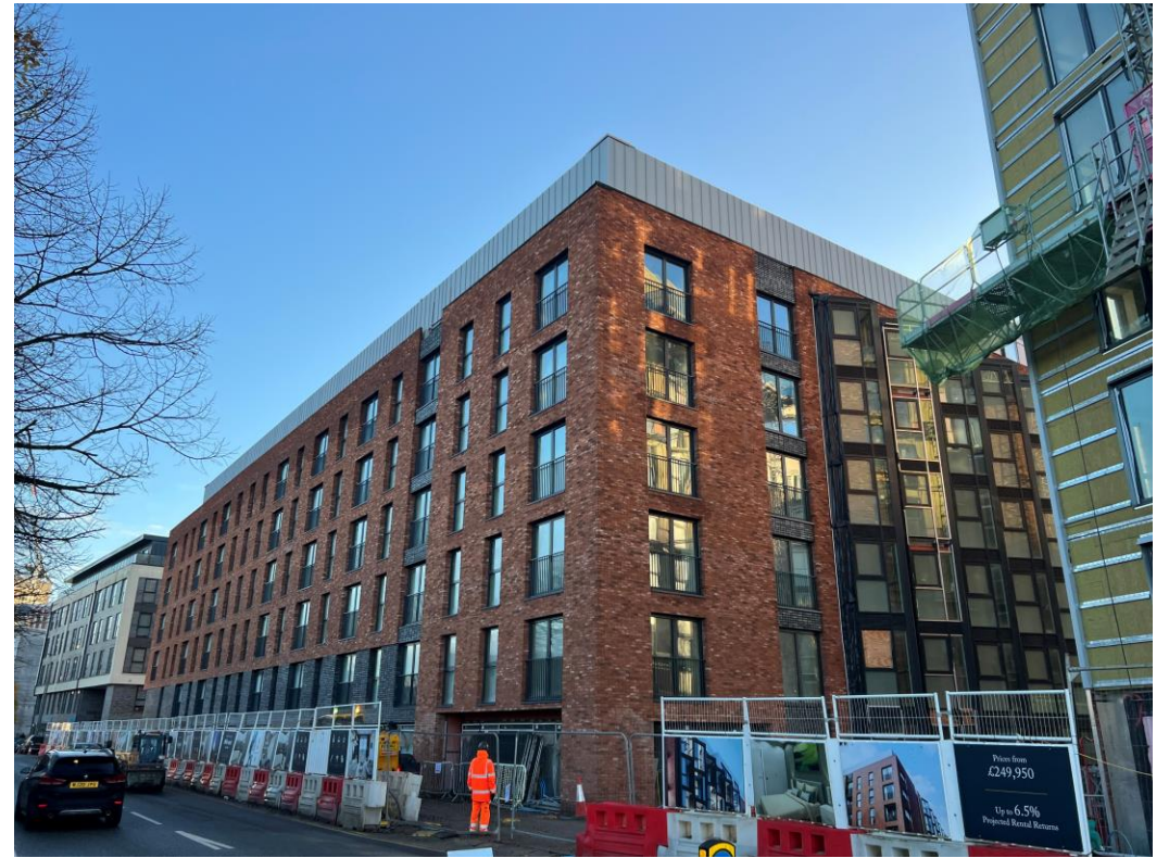
Ordsall Lane site view
