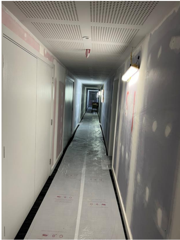
Level 3 – corridor carpet
