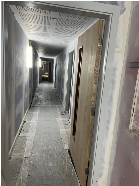
Level 6 – corridor door installed
