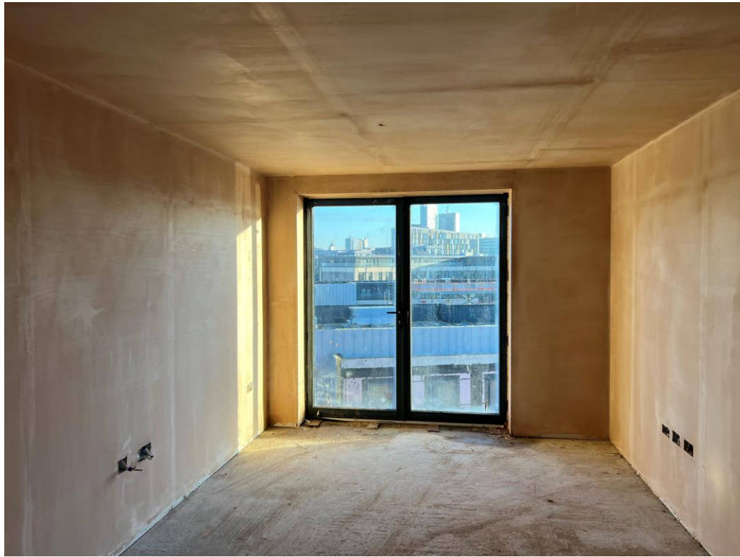
Level 8 – Hoist apartment plaster skim finish
