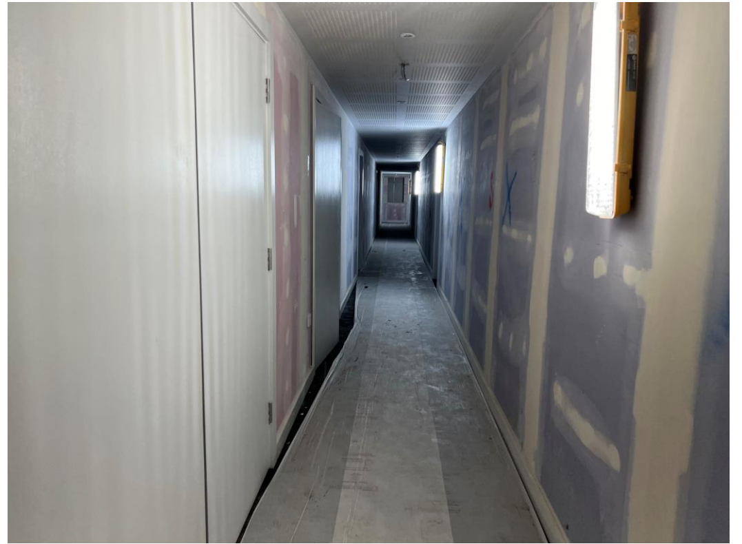
Level 6 – corridor carpet
