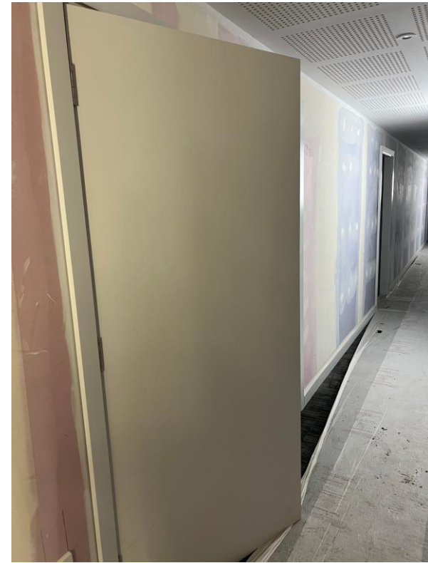
Level 6 – services cup'd doors painted
