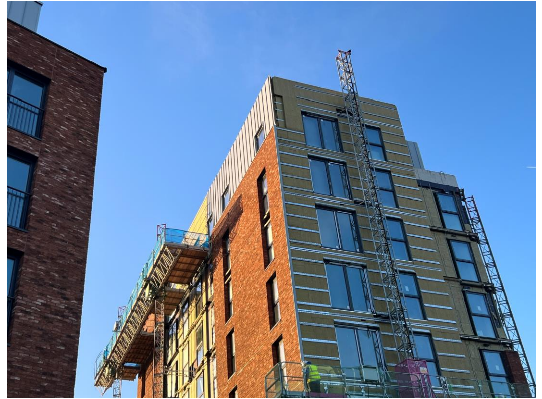
Ordsall Lane site view
