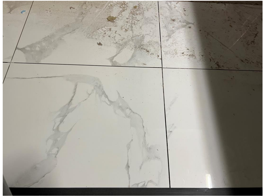
Level 3 – floor tiling lift lobby
