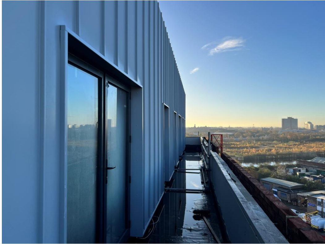
Block A wall cladding
