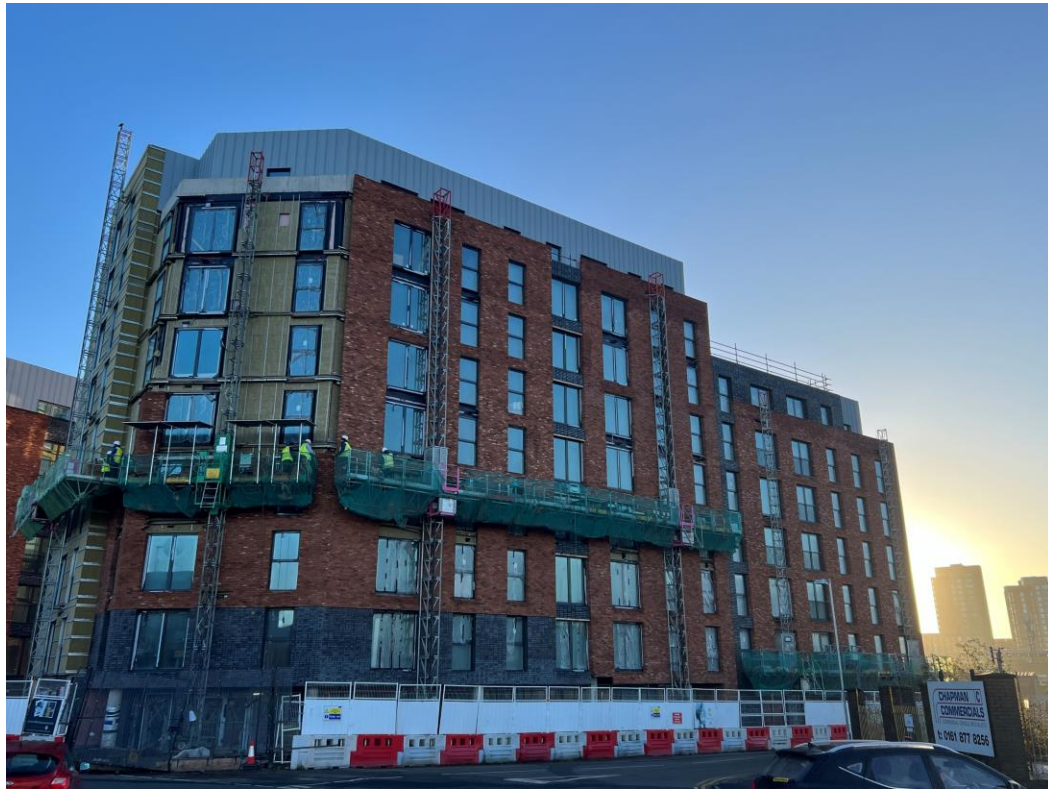
Worrall Street site view
