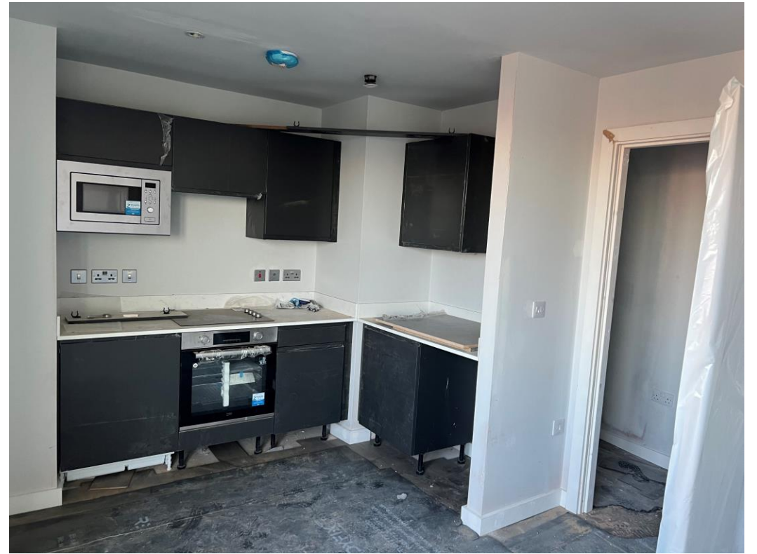
Level 8 – Kitchen units & worktops installed
