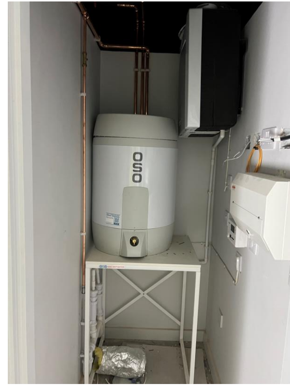
Level 3 – 2 nd fix mechanical & electrical
