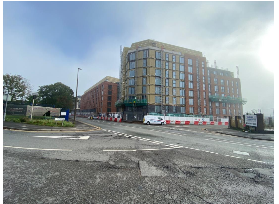
Ordsall Lane site view
