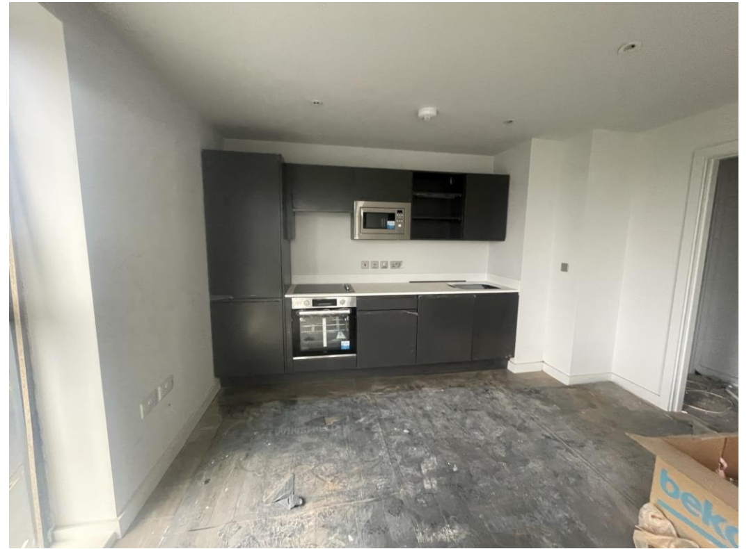
Level 7 – Kitchen units & appliance installed
