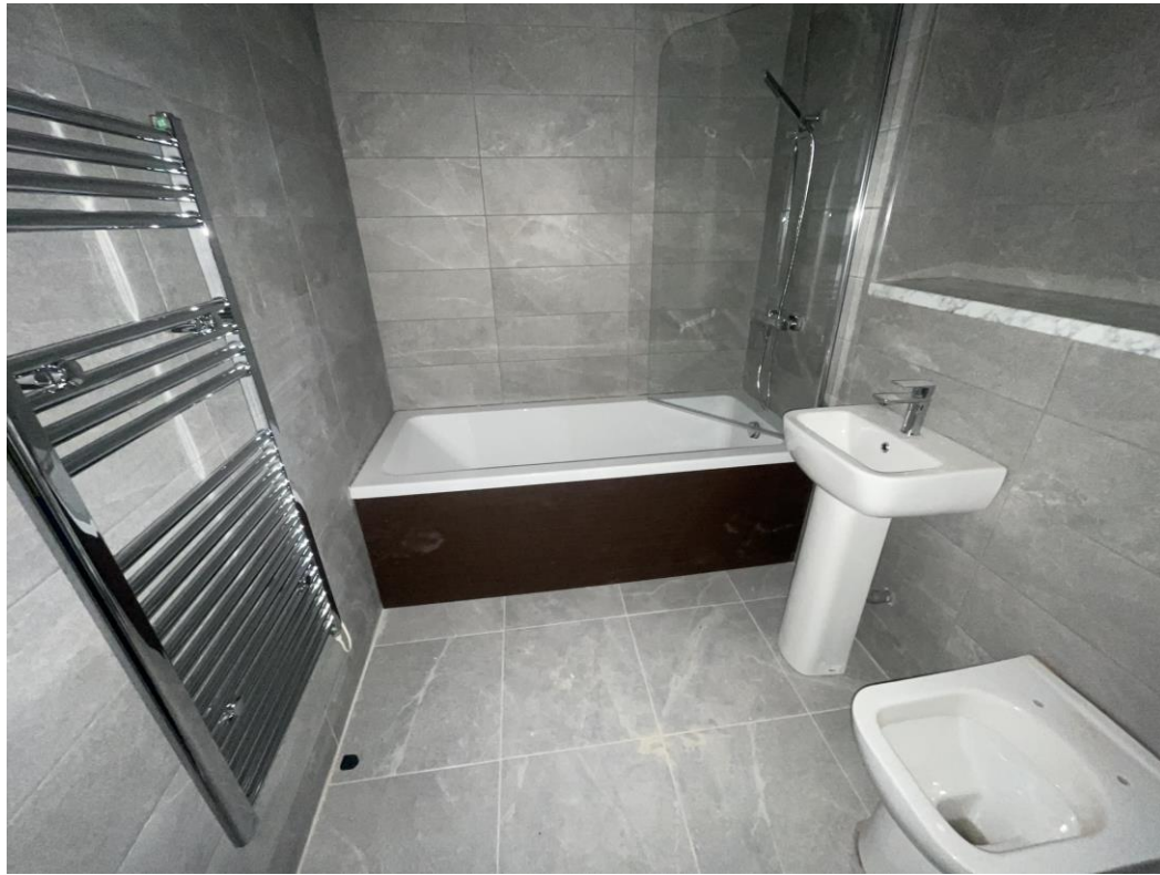
Level 6 – Sanitary appliances installed
