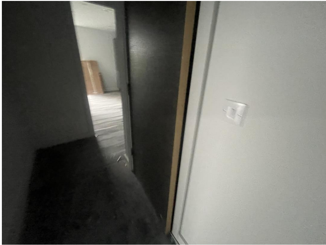
Level 2 – Internal doors installed
