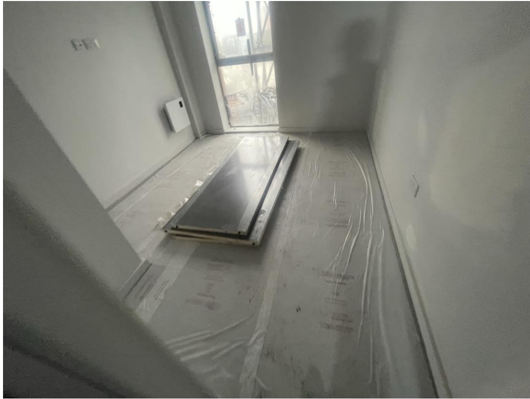
Level 2 – Internal doors loaded
