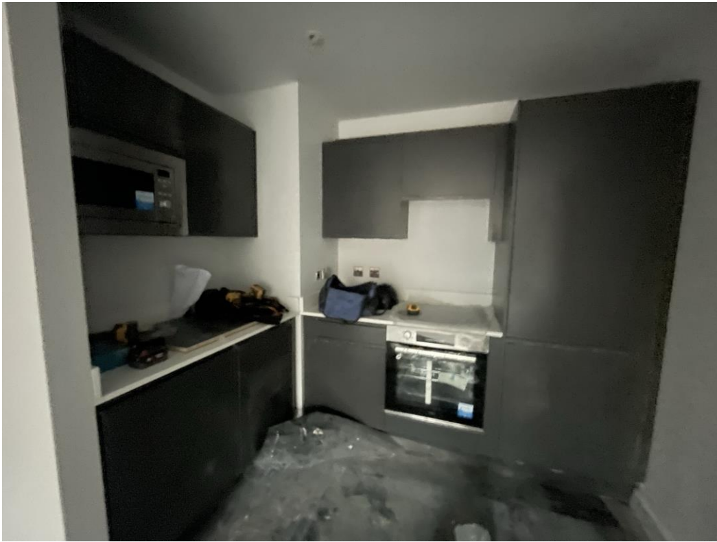
Level 4 – Kitchen units & worktop installed
