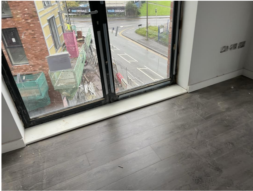
Level 3 – Timber window board installed
