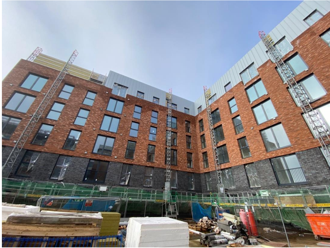
Block B – Cladding & brickwork
