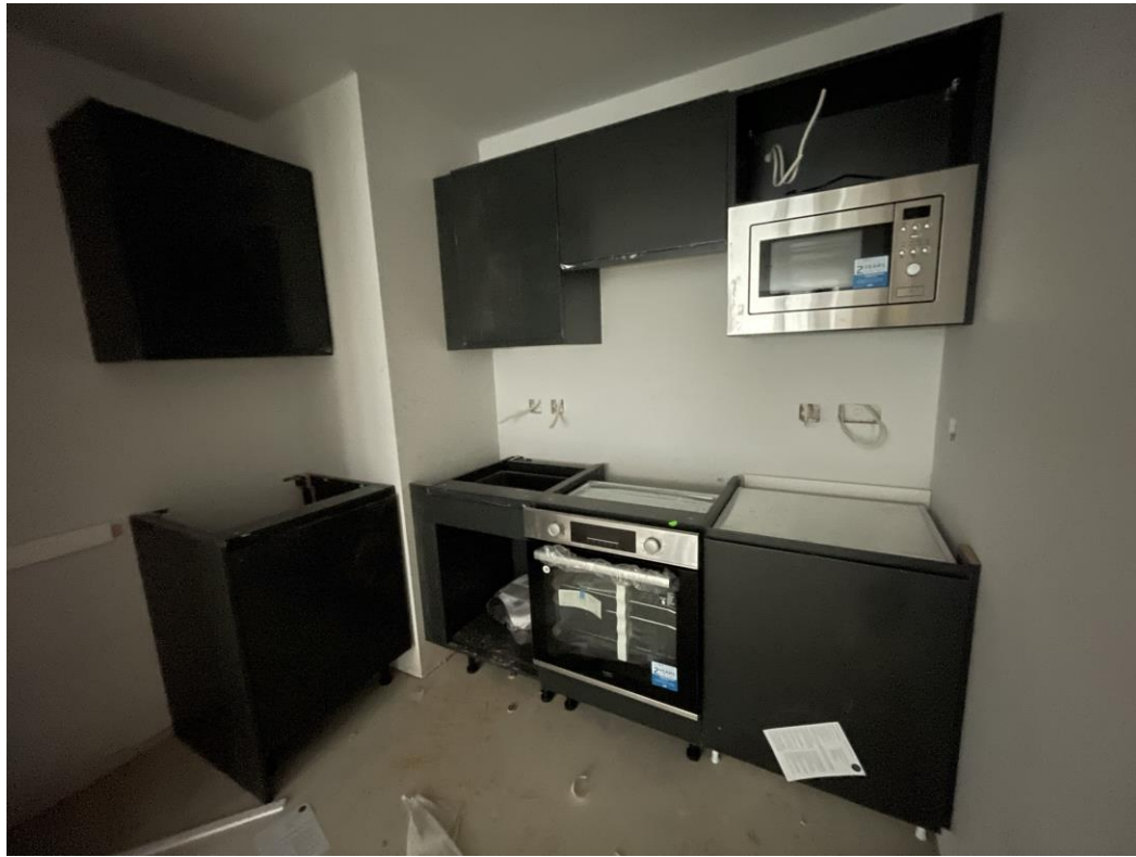
Level 1 – Kitchen units commenced
