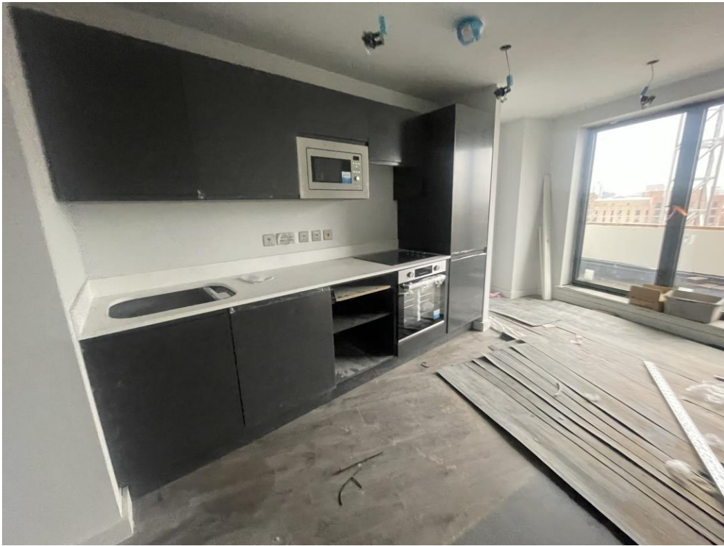
Level 6 – Kitchen units & appliance installed
