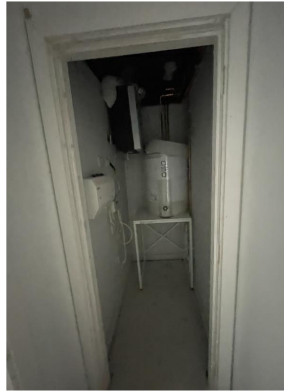
Level 3 – 2 nd fix mechanical & electrical
