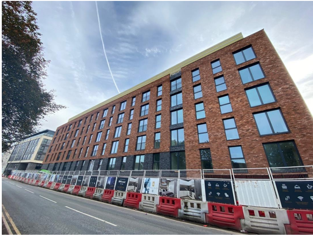
Ordsall Lane site view
