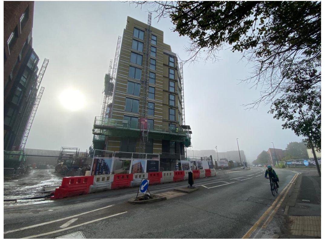
Ordsall Lane site view
