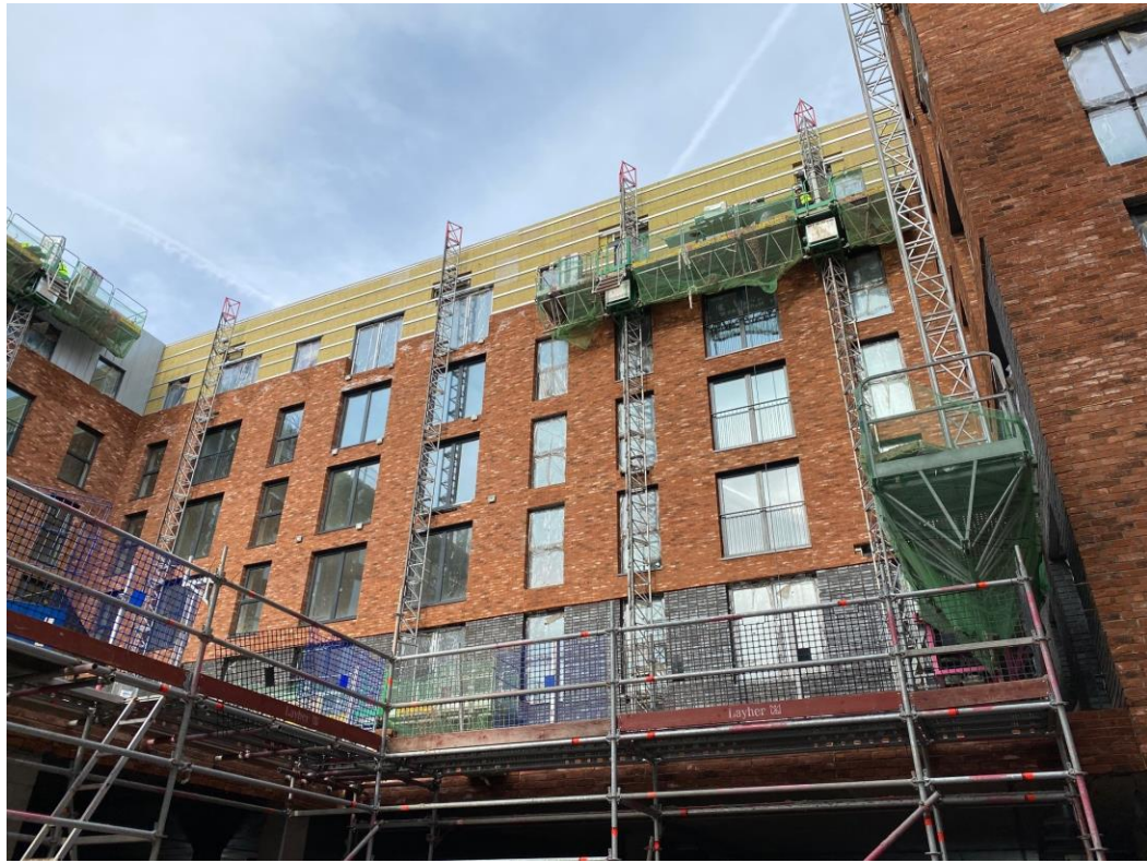
Block B – Brickwork
