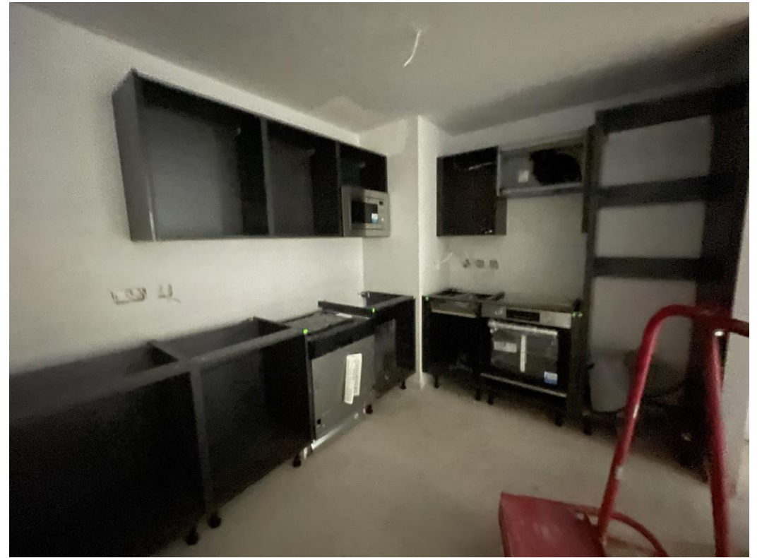
Level 1 – Kitchen units commenced
