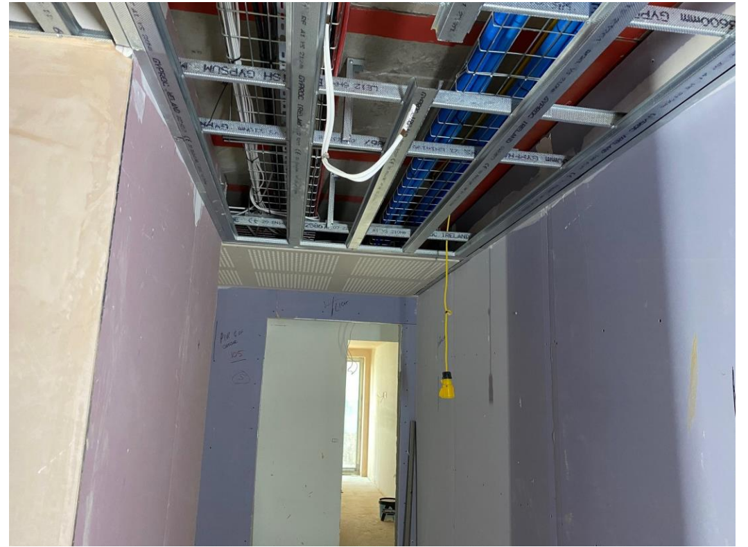
Level 1 – Corridor ceiling grid erected
