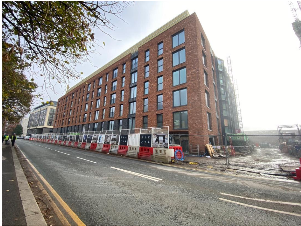
Ordsall Lane site view
