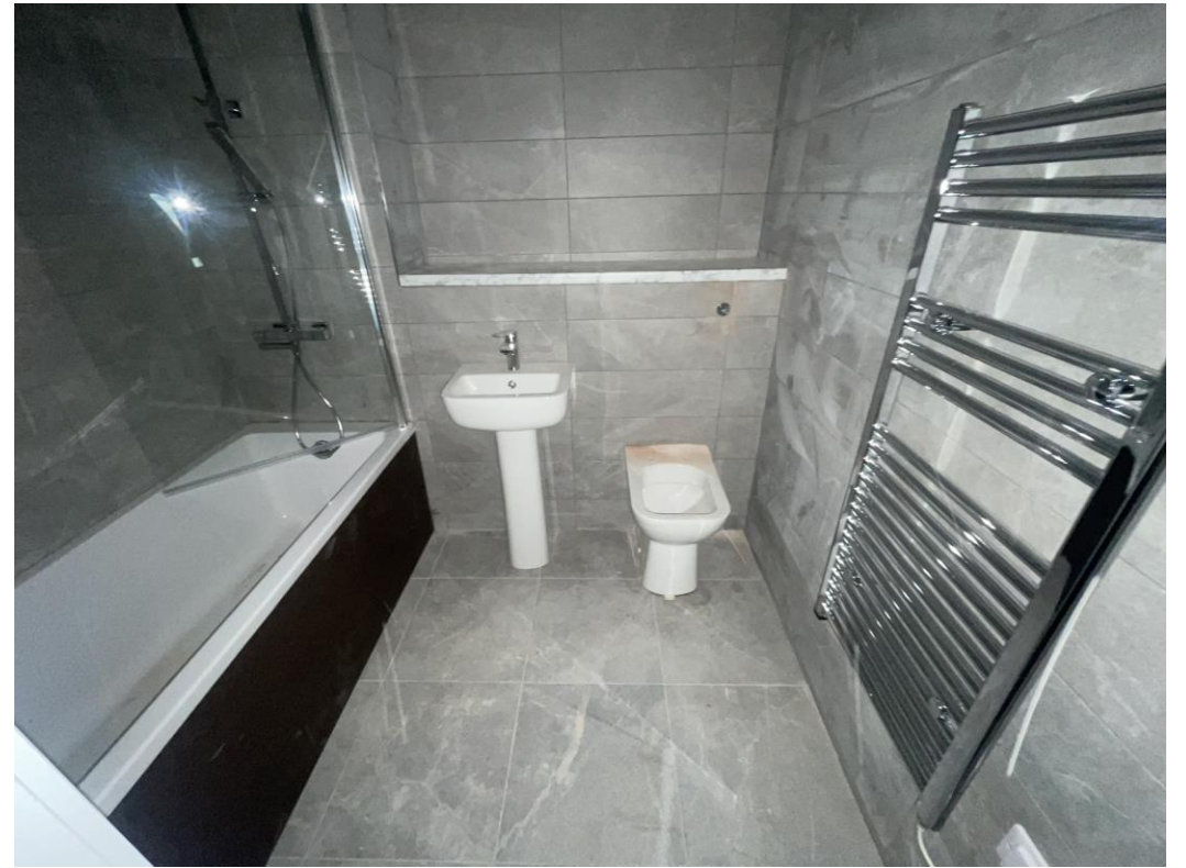
Level 6 – Sanitary appliances installed
