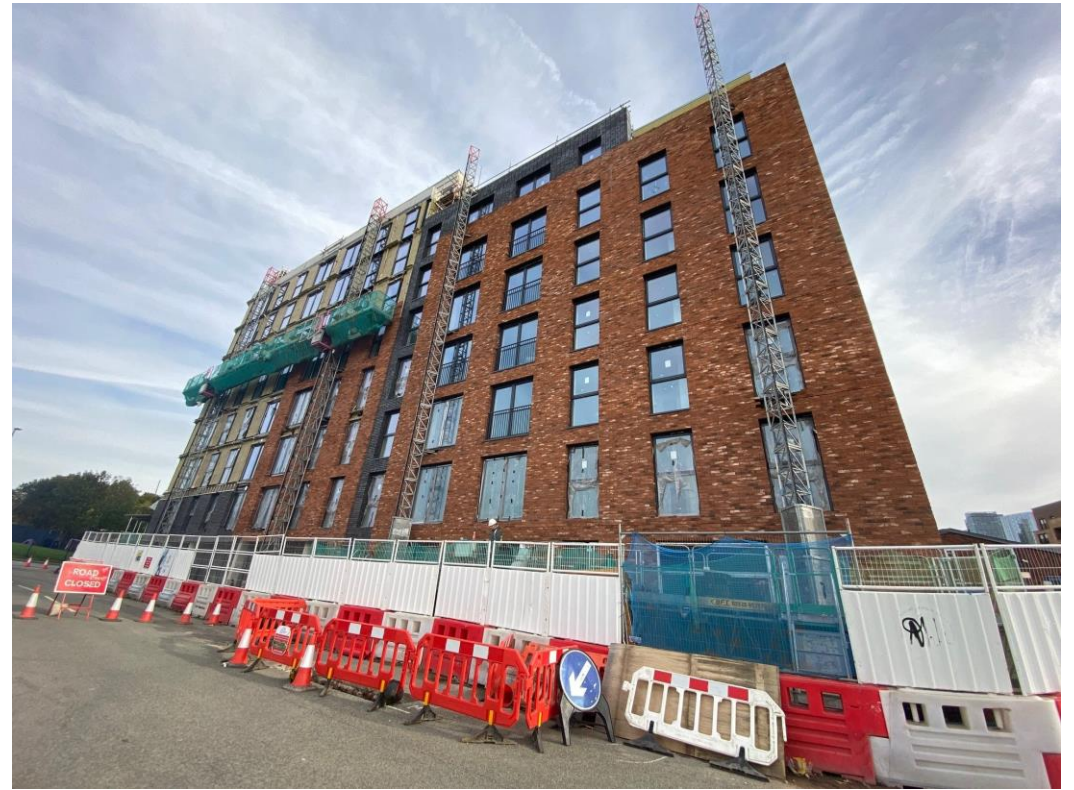
Ordsall Lane site view
