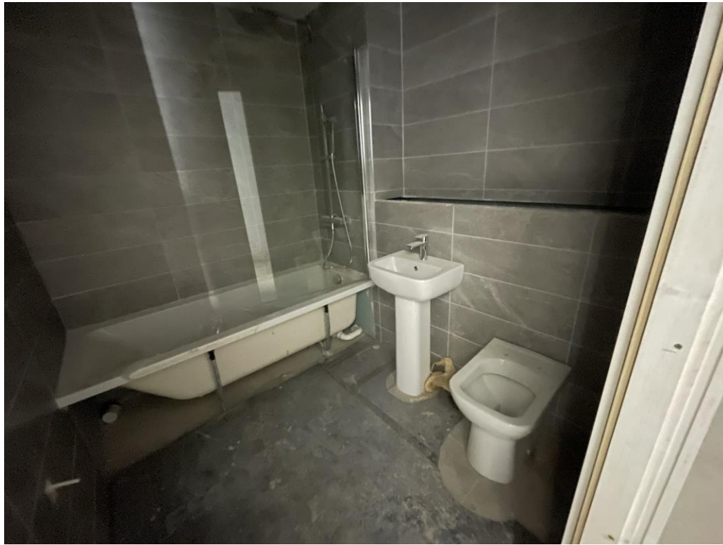
Sanitary appliances installed
