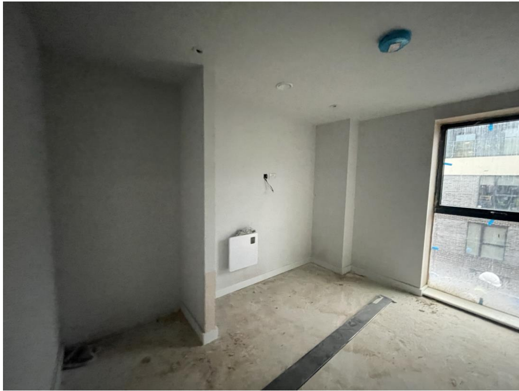
Level 5 – Decorations commenced walls and ceilings
