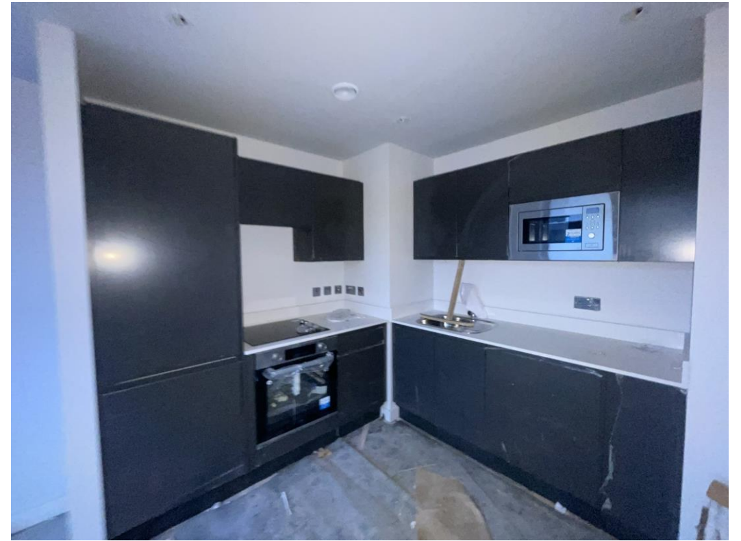
Level 6 – Kitchen units and appliances installed
