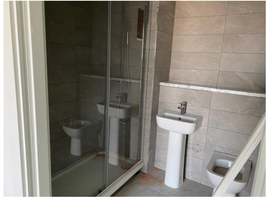
Sanitary appliances installed
