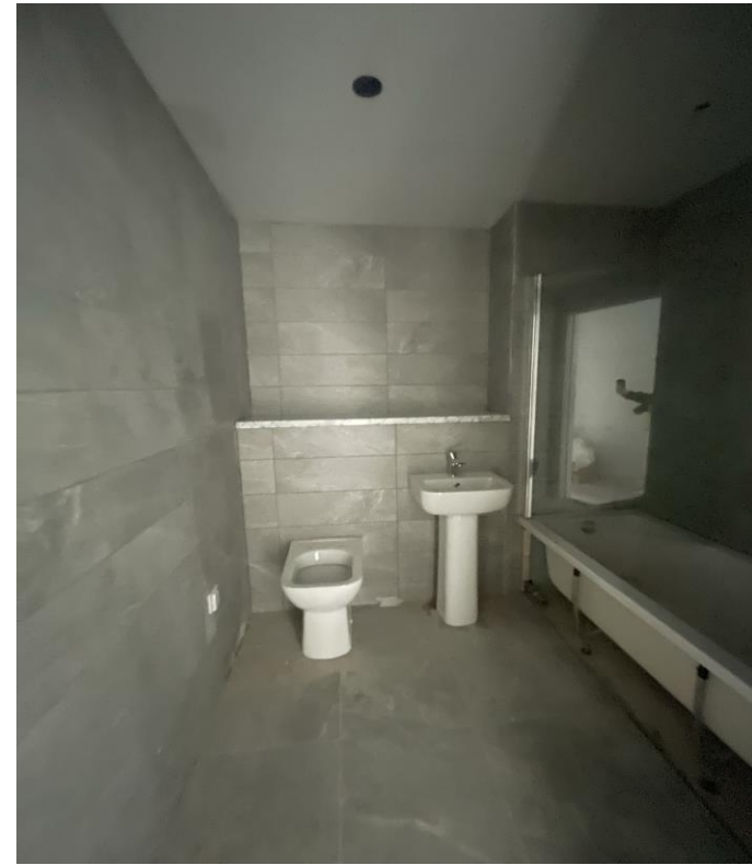
Level 6 – Sanitary appliances installed
