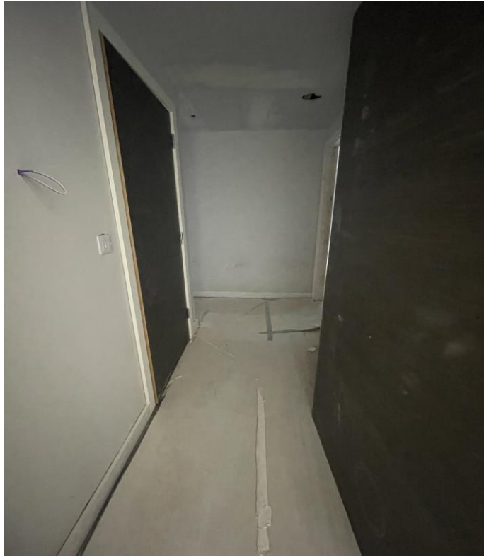
Level 2 – Internal woodgrain door installed
