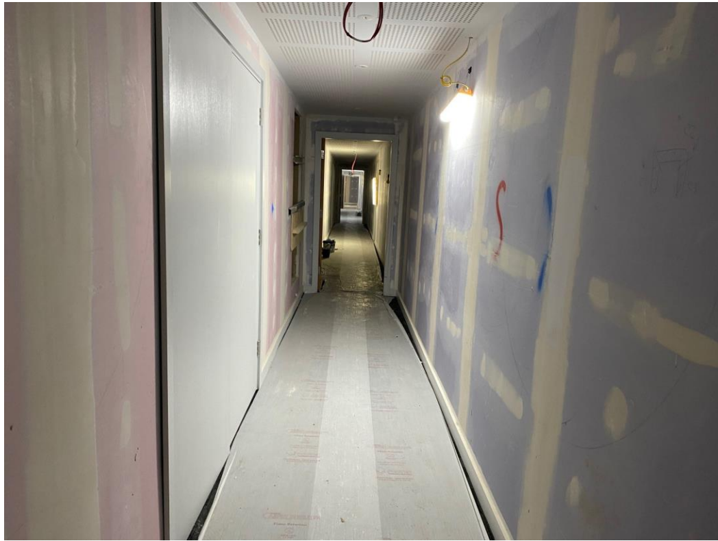
Level 6 – acoustic perforated board to corridor ceiling & fire doors
