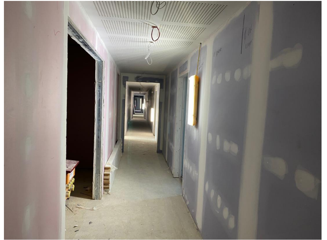
Level 2 – Wall tape & jointing on-going
