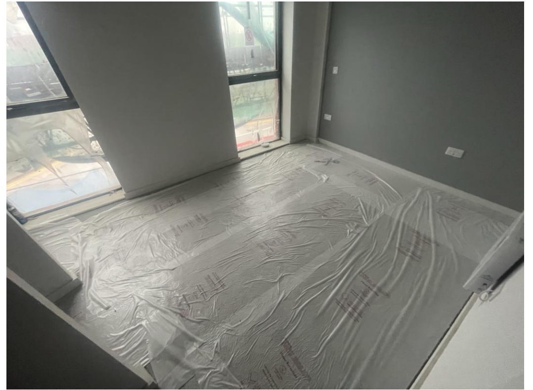
Level 2 – Carpets installed
