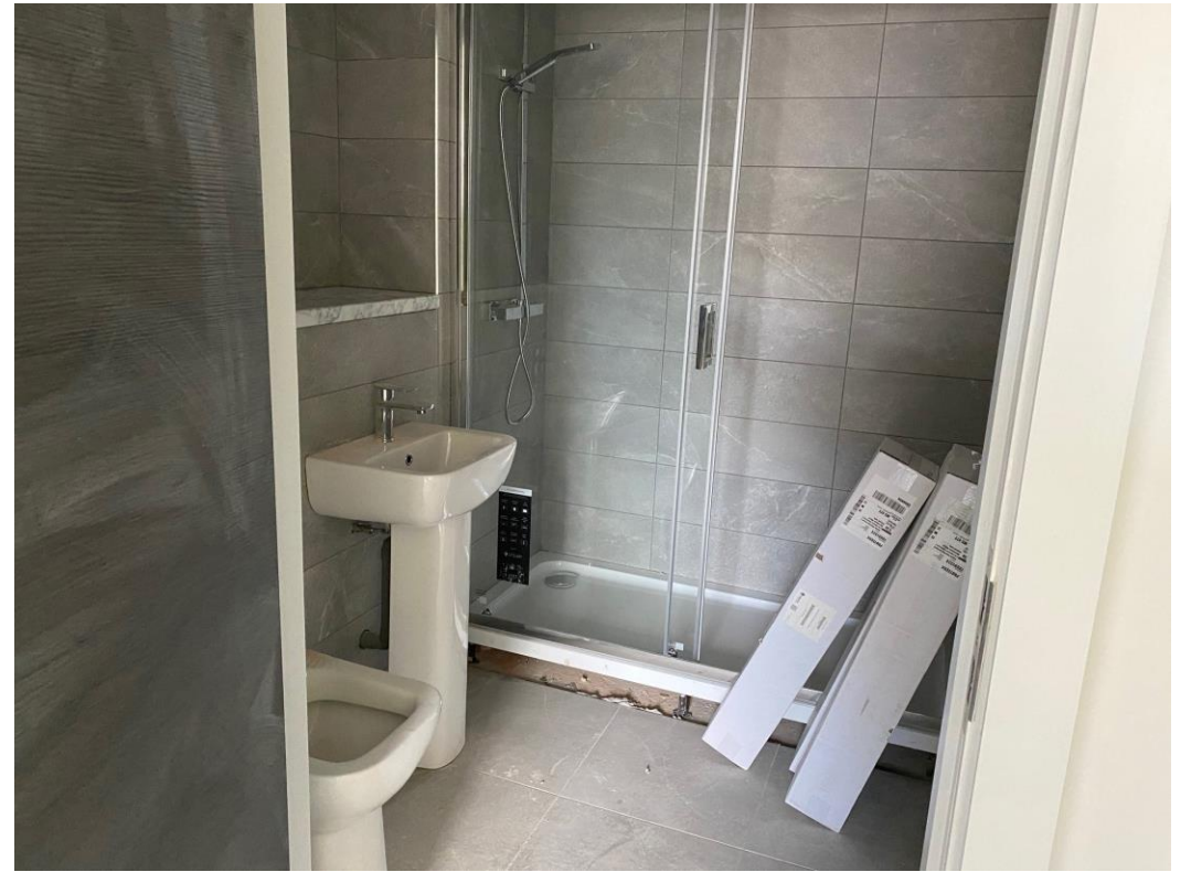
Level 6 – Sanitary appliances installed
