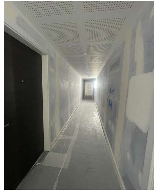
Level 6 – Carpet floor covering
