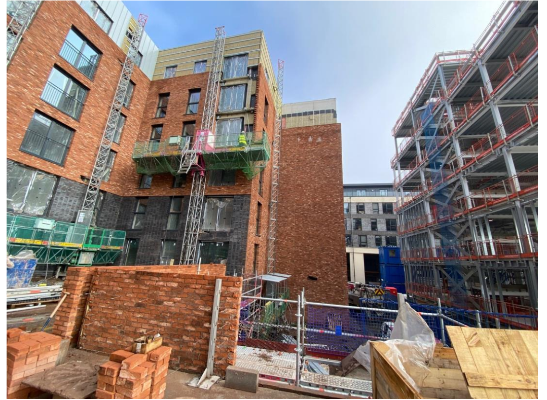
Block B – Cladding & brickwork
