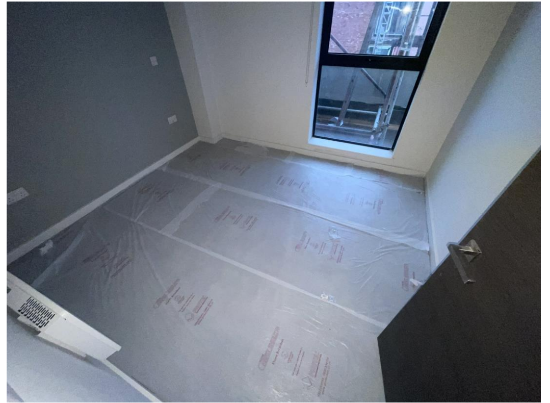
Level 6 – Carpet floor covering
