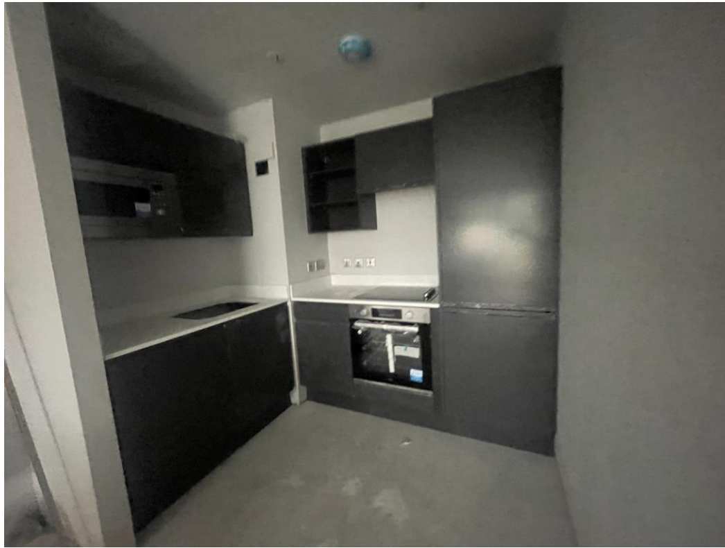
Level 7 – Kitchen units & appliance installed
