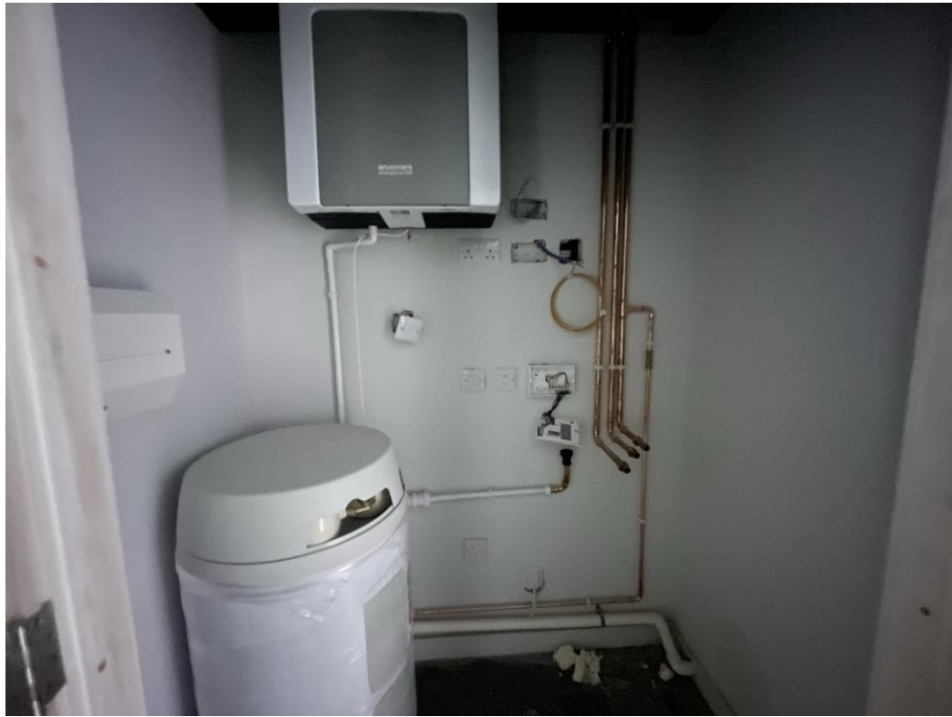
Level 3 – 2 nd fix mechanical & electrical
