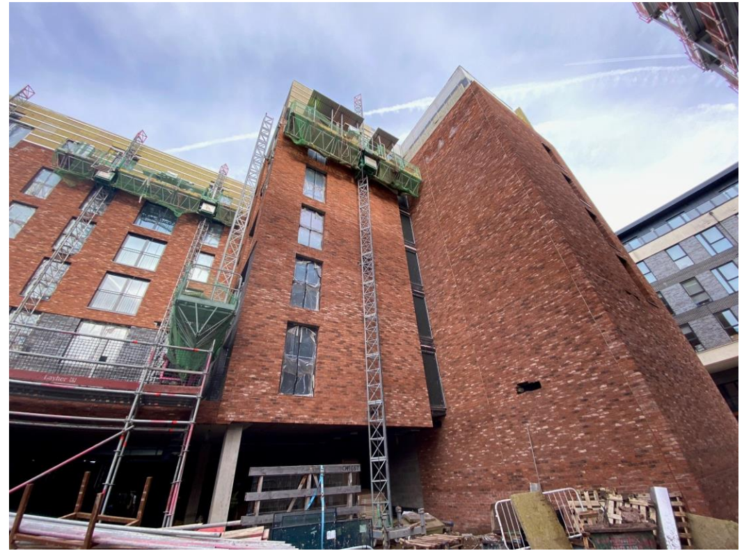
Block B – Brickwork
