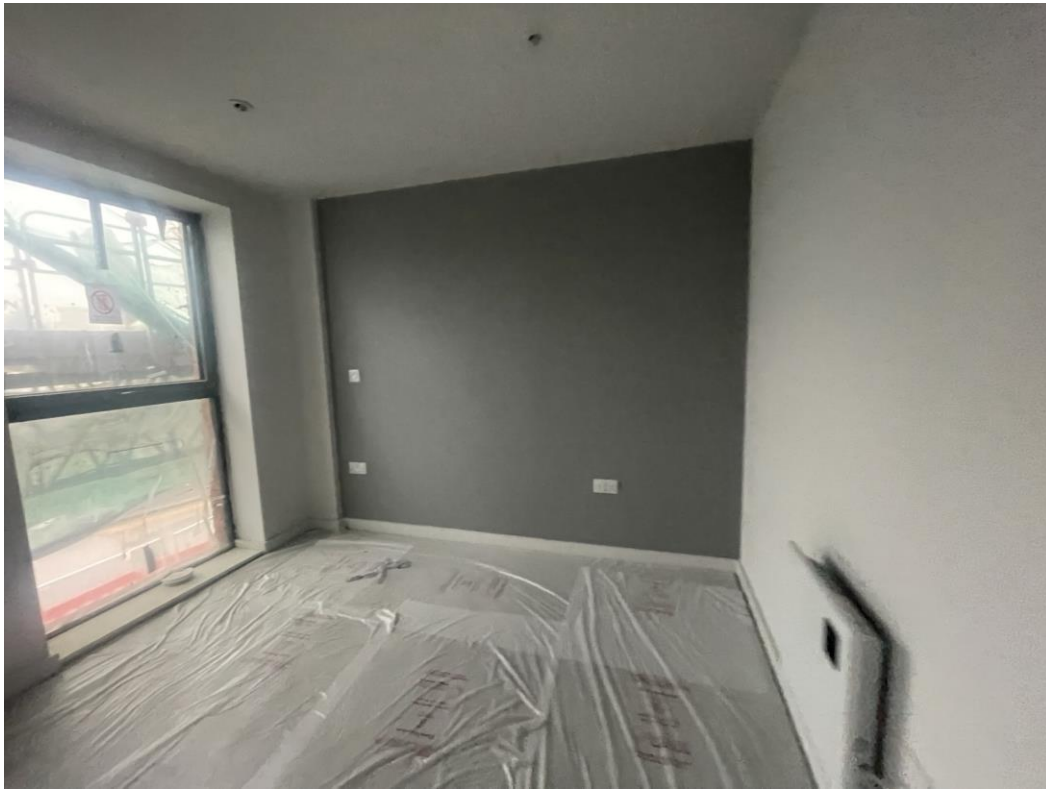
Level 1 – Bedroom finishes
