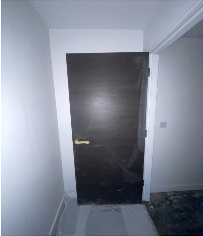
Level 6 – Internal woodgrain door installed
