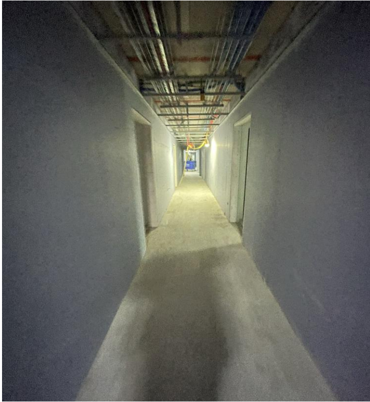
Level 1 – Boarding of corridor walls
