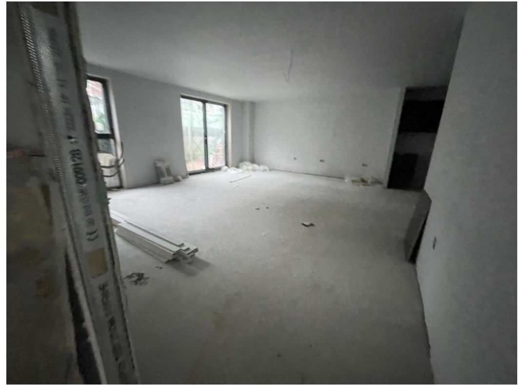
Ground Level – mist coat decoration
