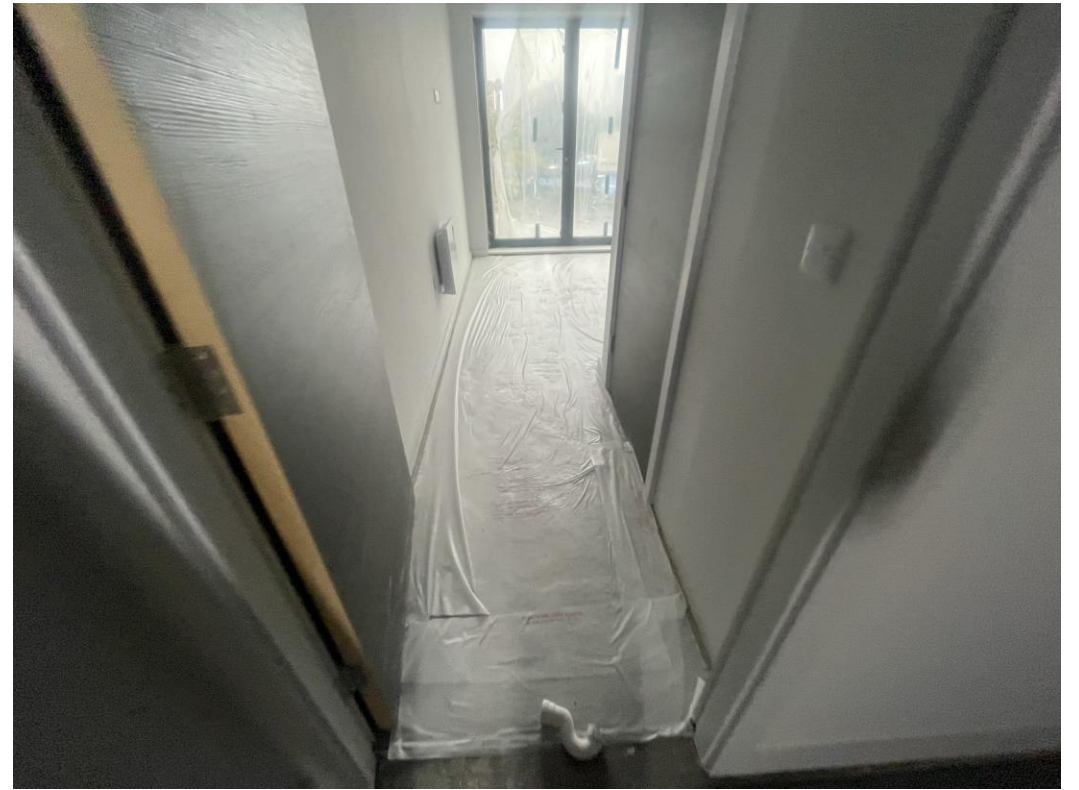
Level 2 – Internal doors installed
