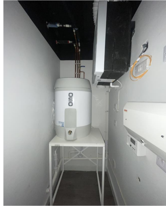
Level 5 – 2 nd fix mechanical & electrical
