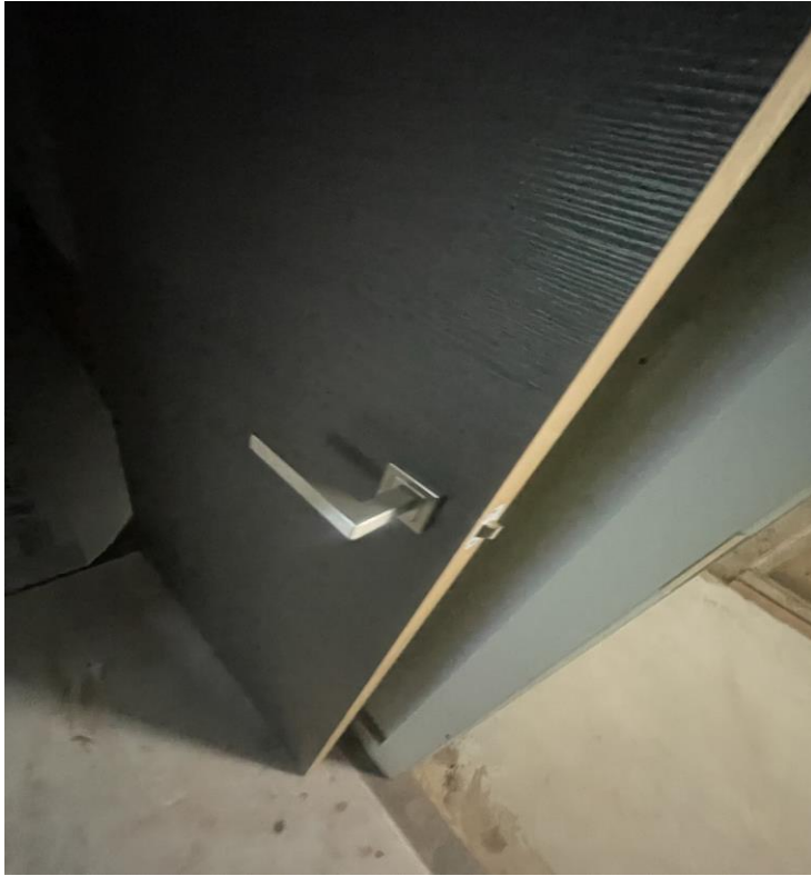
Level 1 – Internal doors & ironmongery installed
