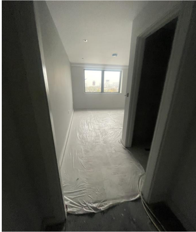
Level 6 – carpet floor covering
