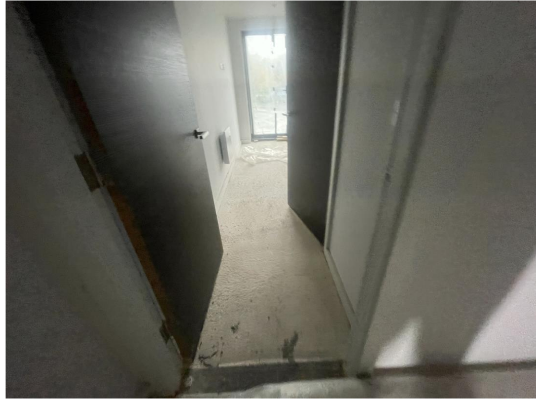
Level 1 – Internal doors & ironmongery installed
