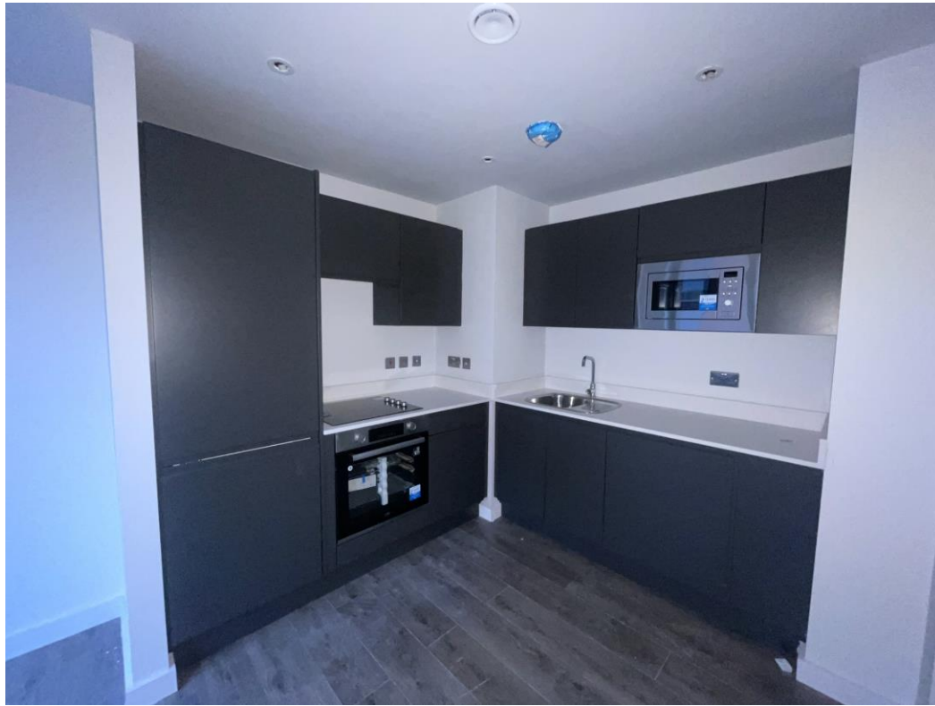
Level 6 – Kitchen units and appliances installed
