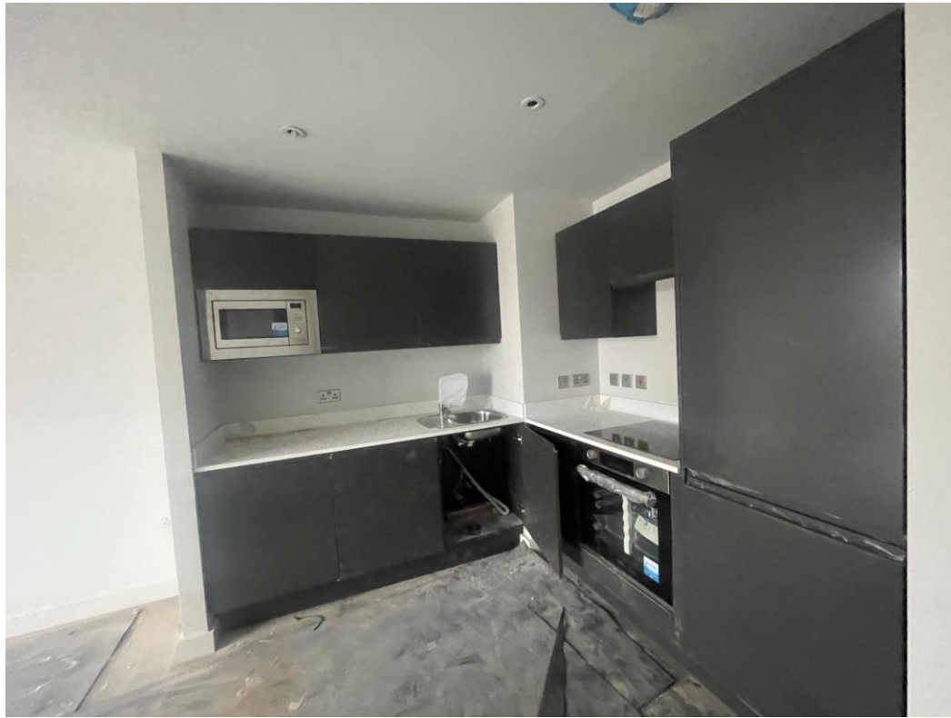
Level 5 – Kitchen units worktop & appliances installed
