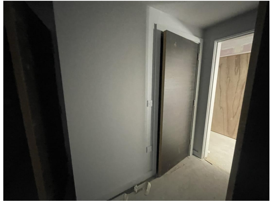
Level 4 – Internal woodgrain door installed
