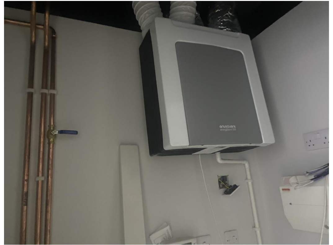
Level 5 – 2 nd fix mechanical
