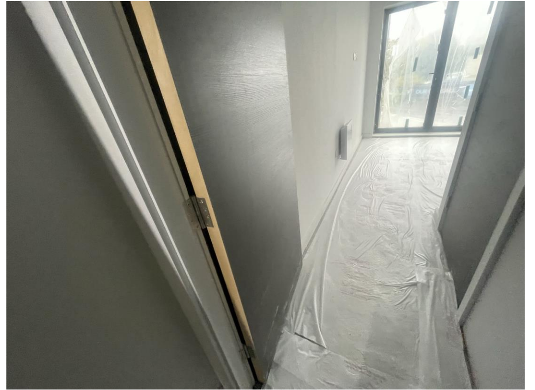
Level 2 – Internal doors loaded
