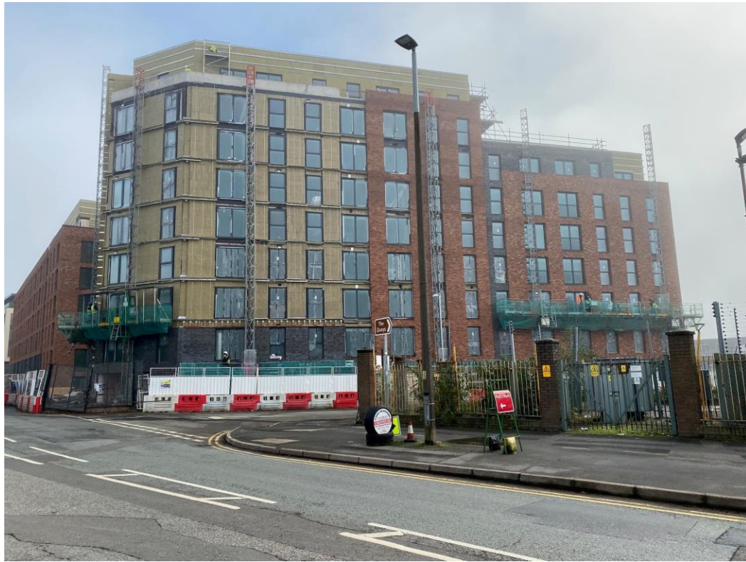
Ordsall Lane site view
