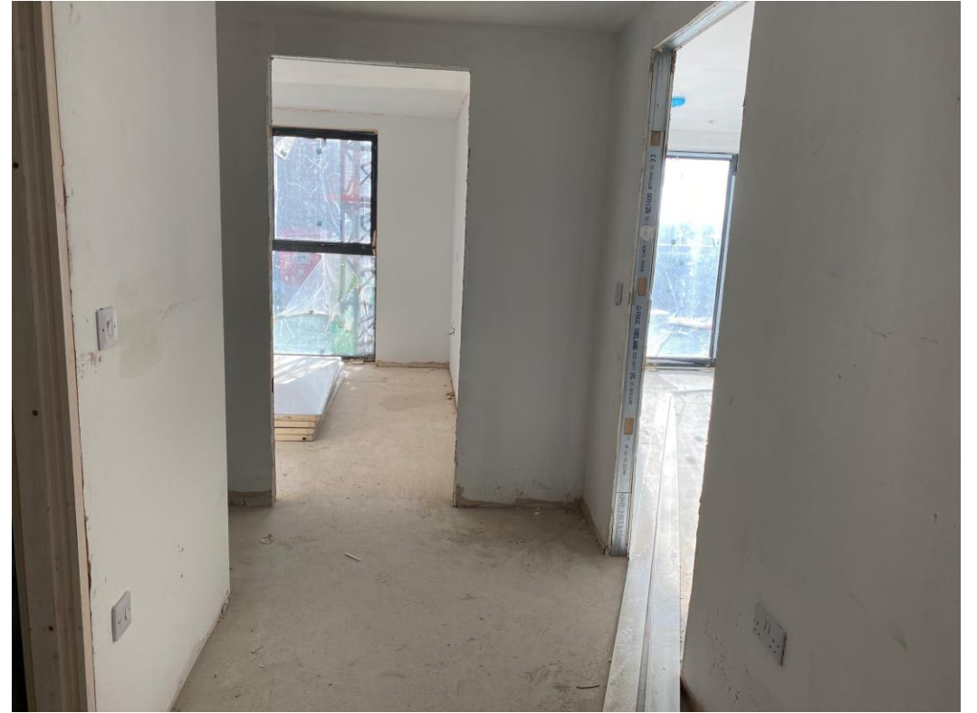
Level 2 – Wall & ceiling decoration commenced
