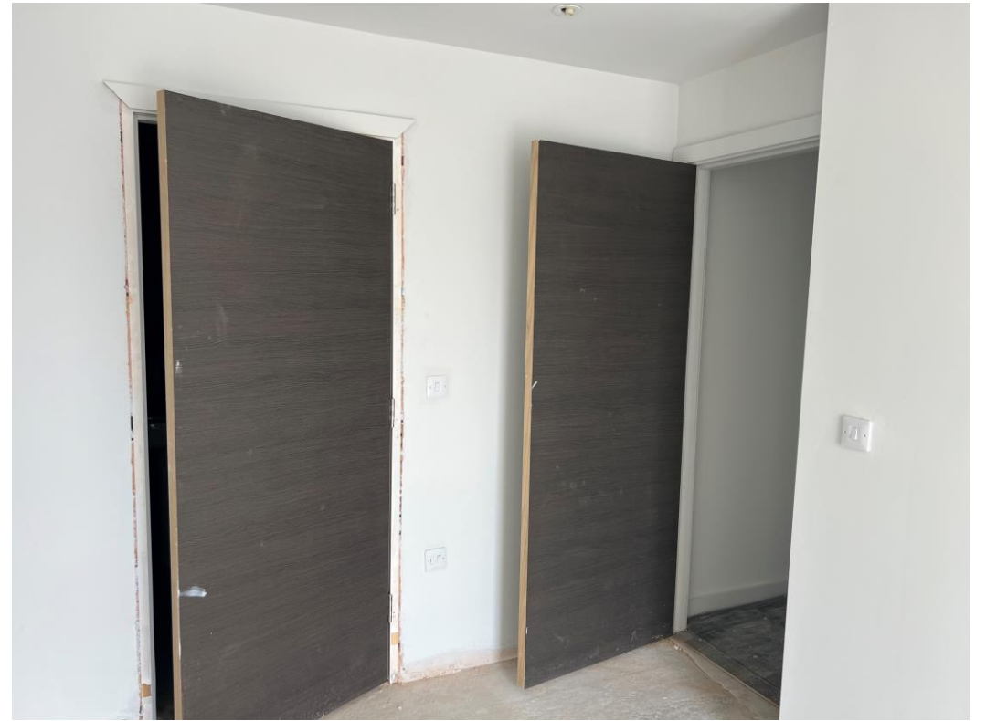
Level 2 – Internal doors installed
