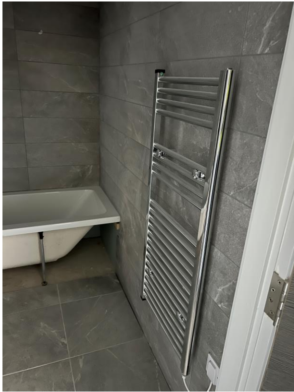
Level 6 – Heated towel rail installed
