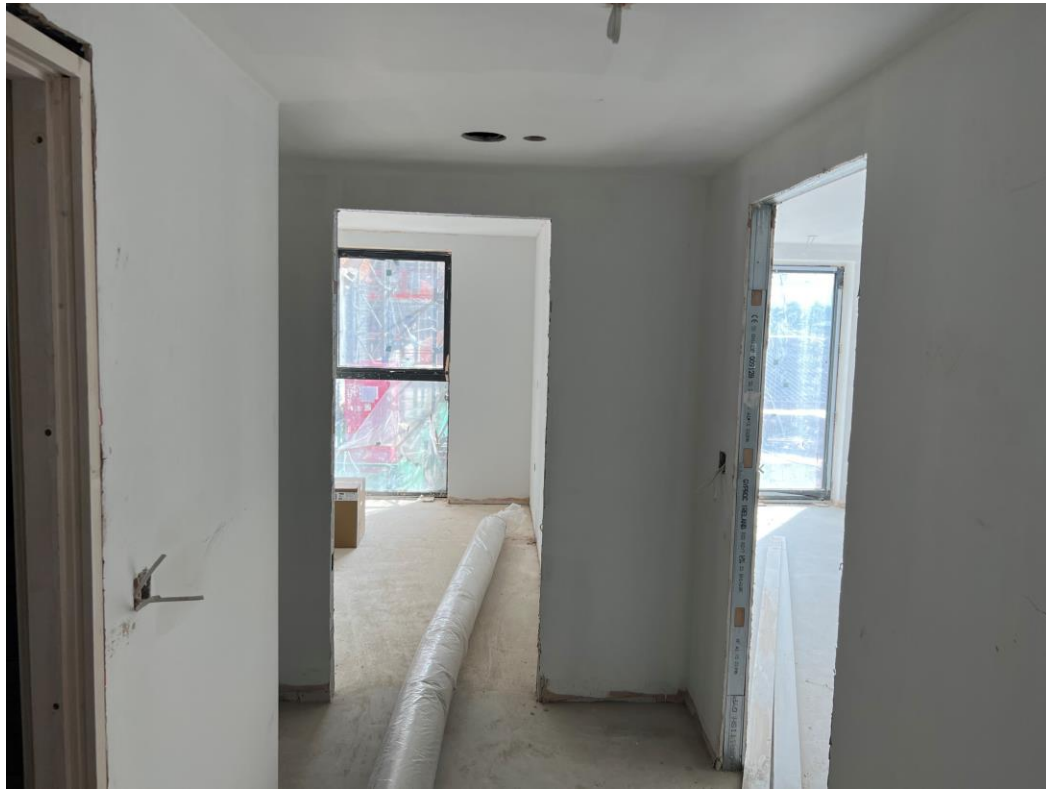
Level 2 – doorframes, skirting and architraves commenced
