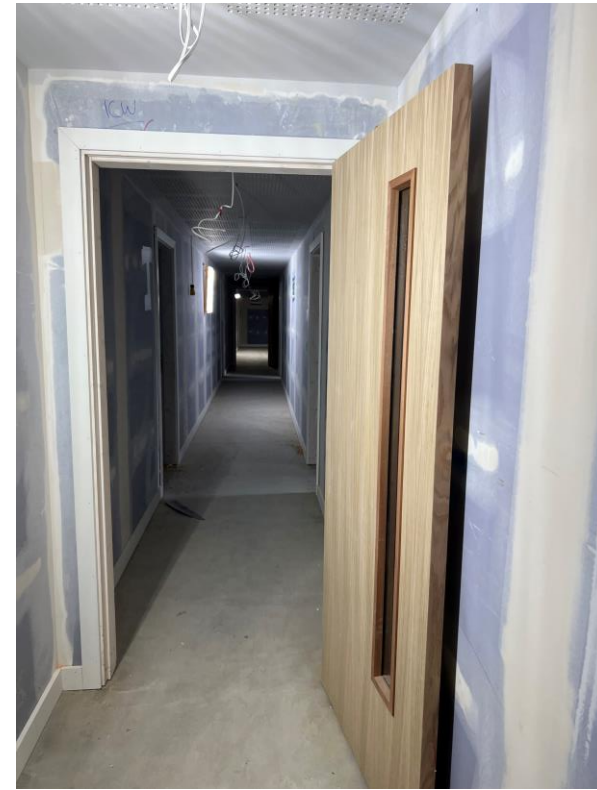
Level 5 – acoustic perforated board to corridor ceiling & fire doors
