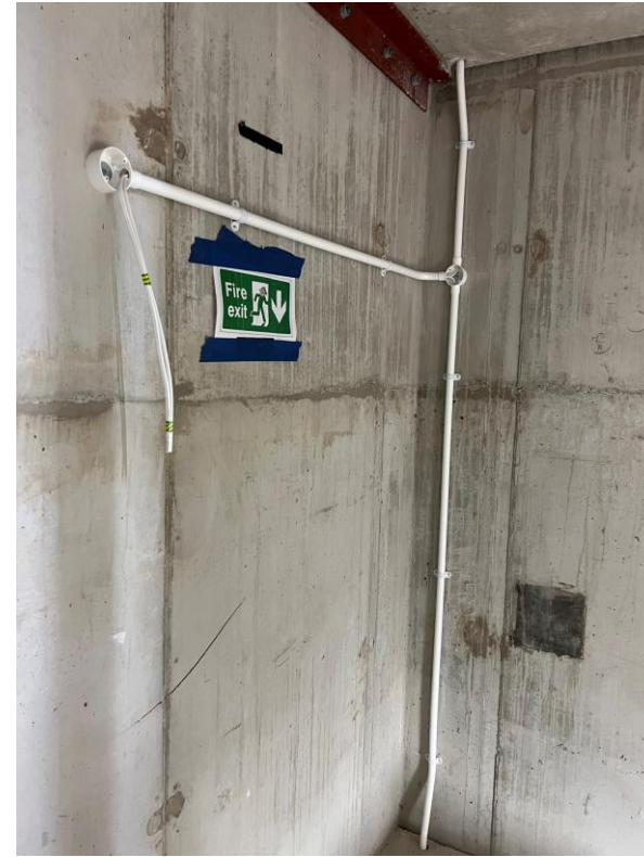
Level 6 – 1 st fix electrical stairwell
