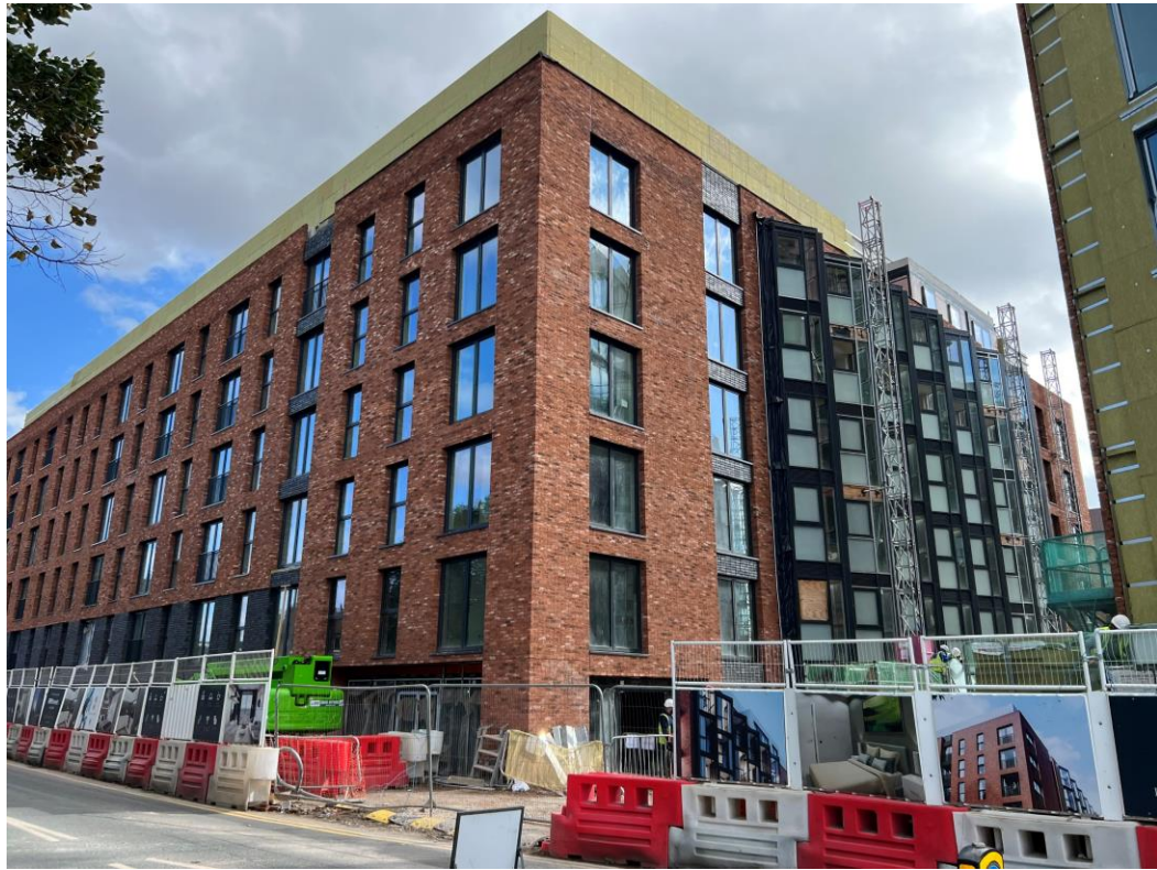
Ordsall Lane site view
