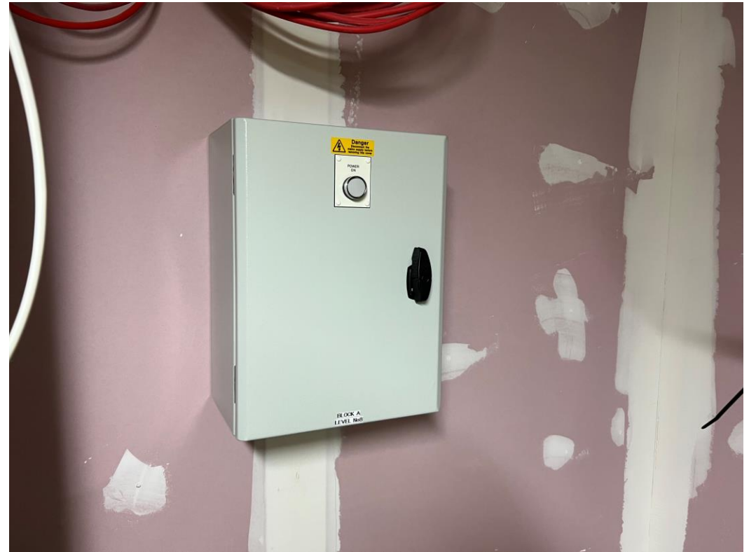
Level 8 – 2 nd fix electrical installation
