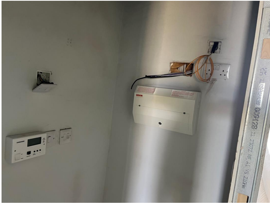
Level 7 – 2 nd fix electrical
