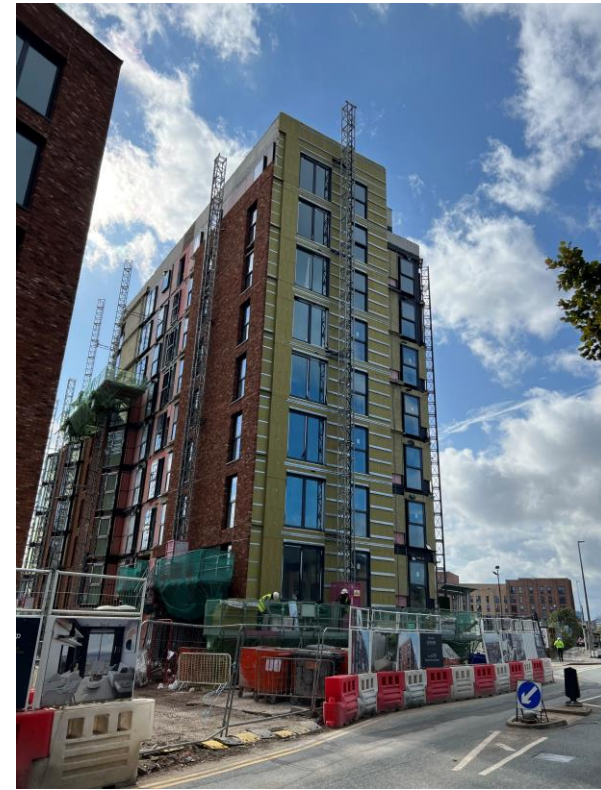
Ordsall Lane site view
