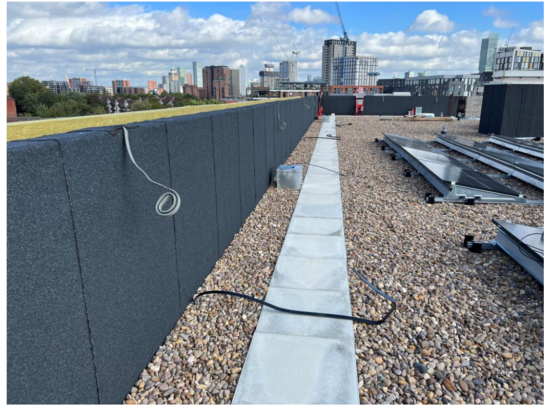
Block B Lightning tape installation
