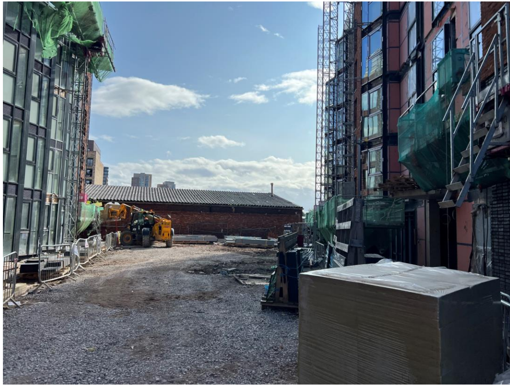
Block A hoist removed
