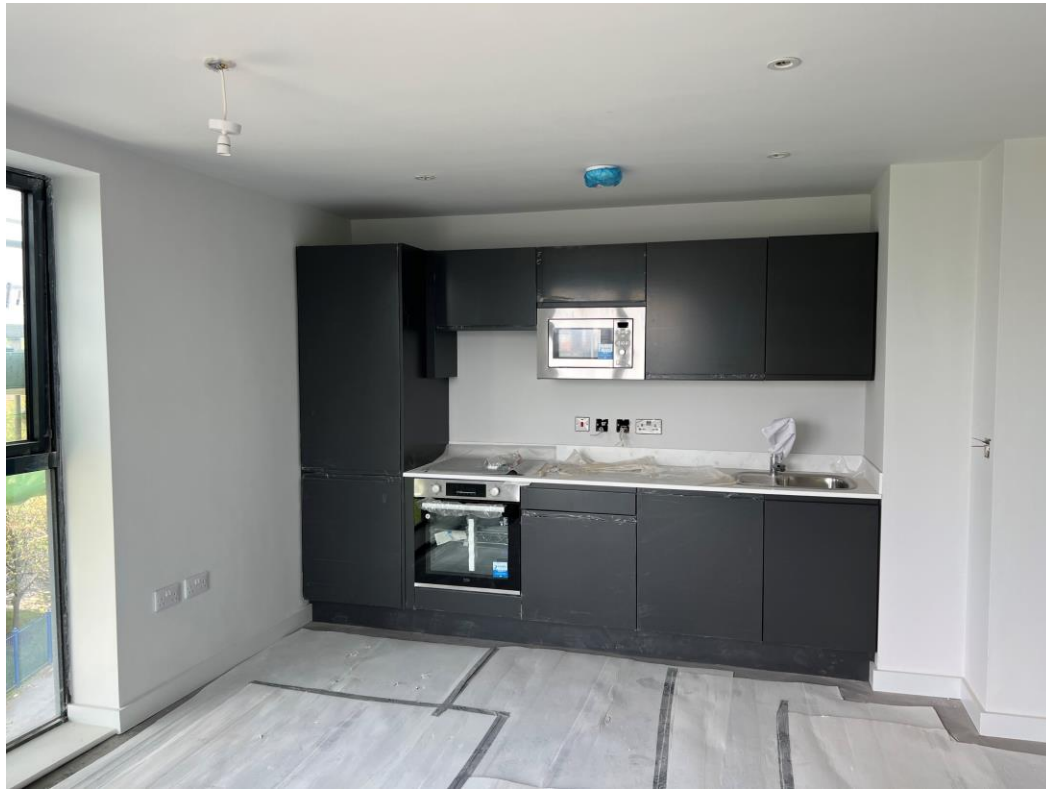
Level 4 – Kitchen complete
