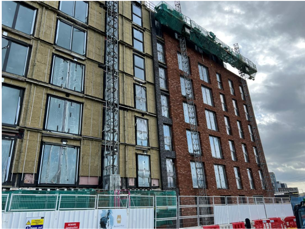
Worrall Street site view
