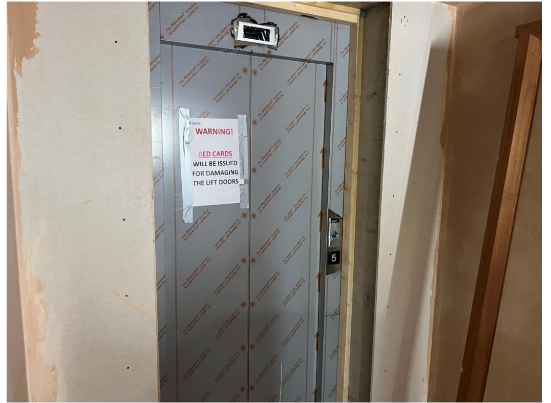
Level 5 – Lift lobby plastered
