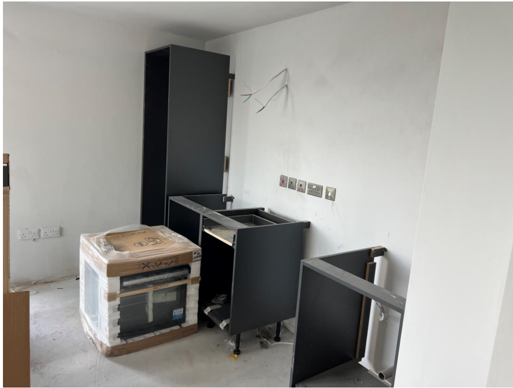
Level 7 – Kitchen units installed
