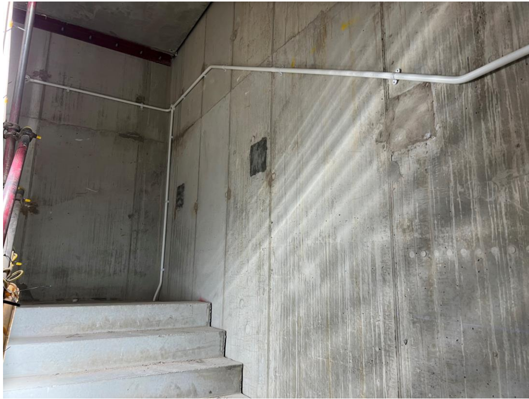
Level 6 – 1 st fix electrical stairwell
