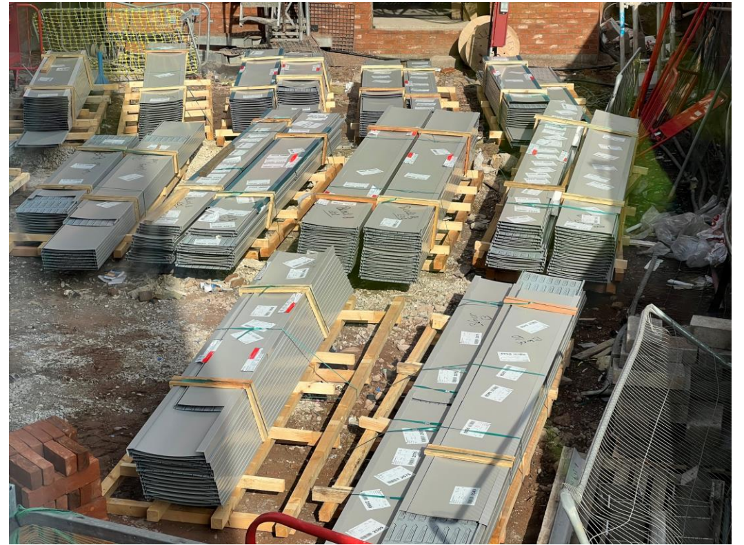
Cladding materials stored
