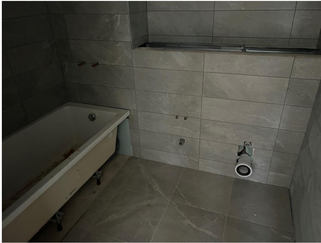
Ground Level – Bathroom wall and floor tiling
