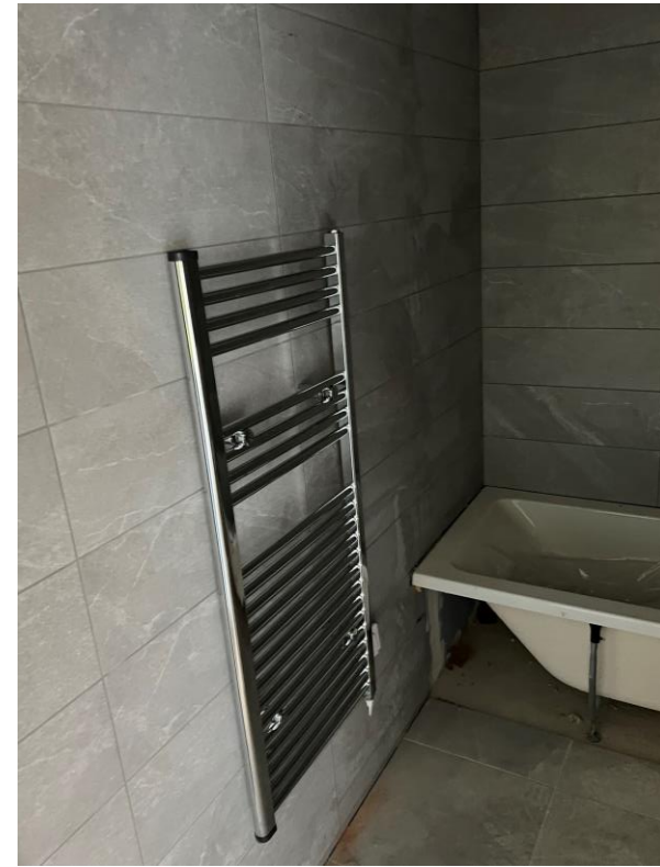
Level 4 – Heated towel rail installed
