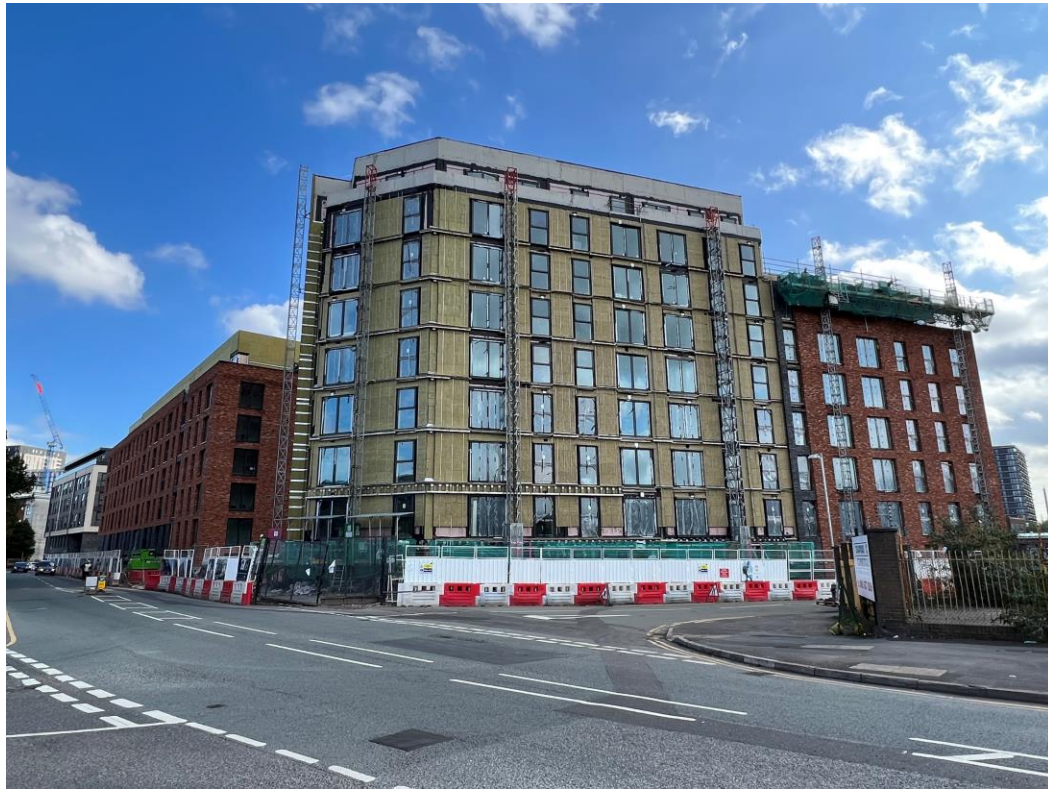
Ordsall Lane site view
