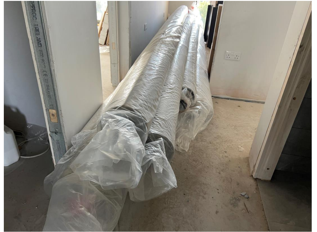
Level 7 – carpet loaded for installation
