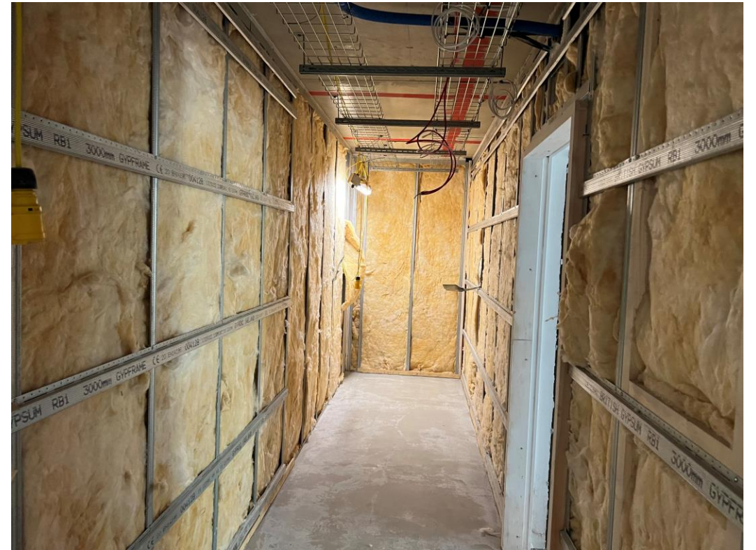
Level 1 – corridors insulated ready for boarding
