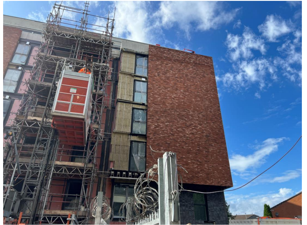
Ordsall Lane site view
