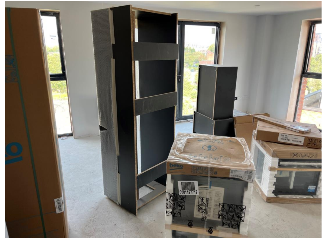
Level 7 – Kitchen units & appliances loaded
