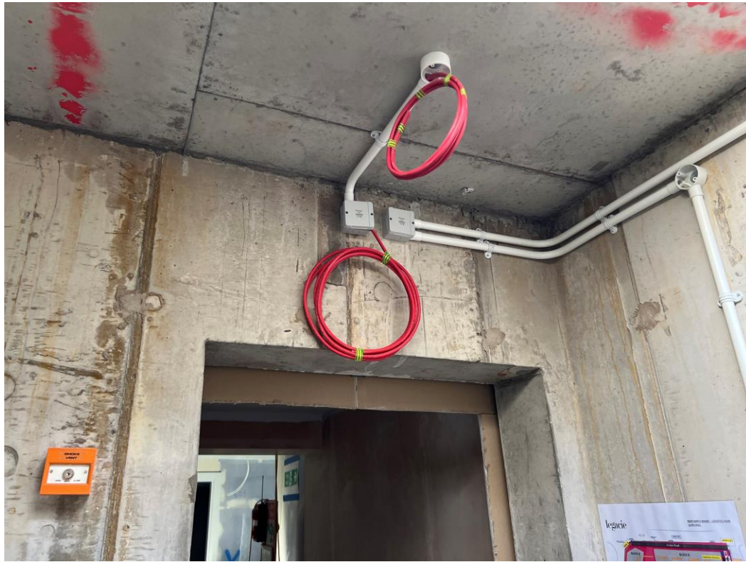
Level 6 – 1 st fix smoke alarm
