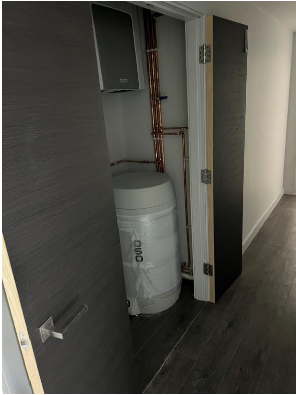
Level 6 – Internal woodgrain doors installed
