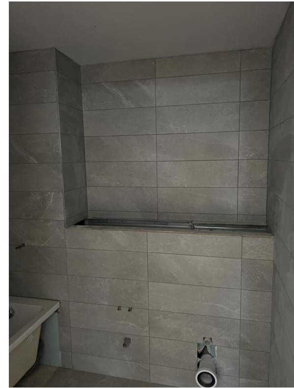
Ground Level – Bathroom wall and floor tiling
