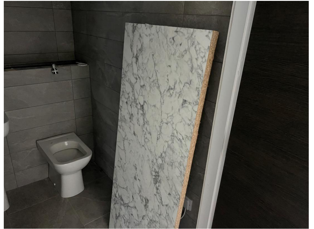
Level 6 – Vanity worktop ready to be installed
