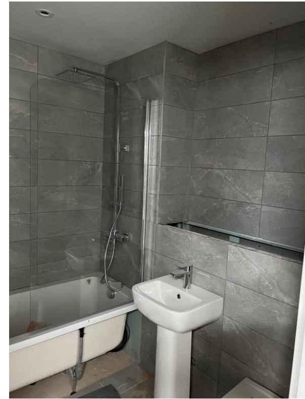
Level 6 – Sanitary appliances installed
