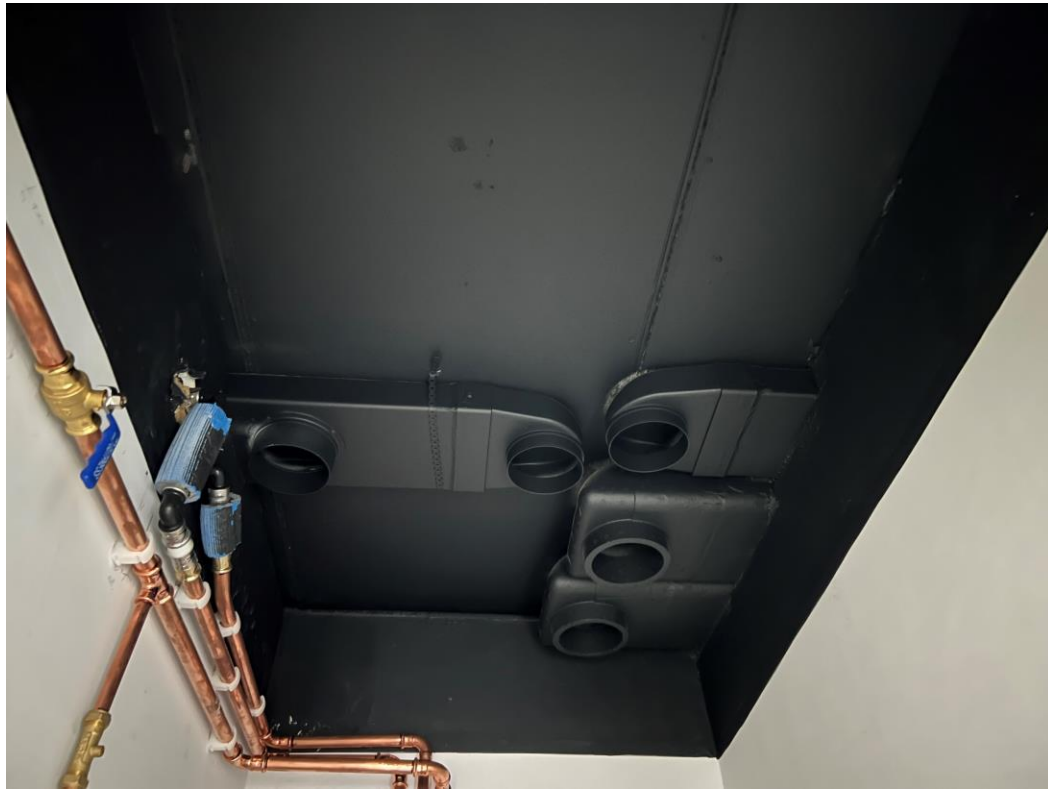
Level 6 – 1 st fix mechanical
