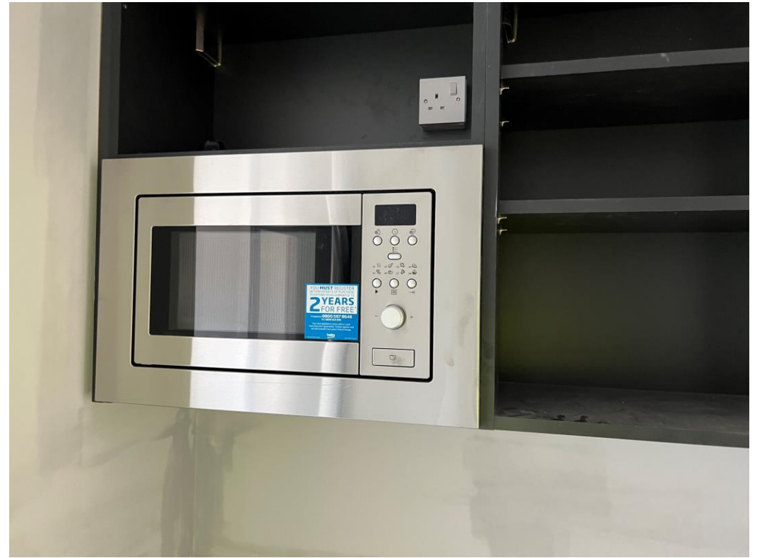
Level 5 – Kitchen appliances installed
