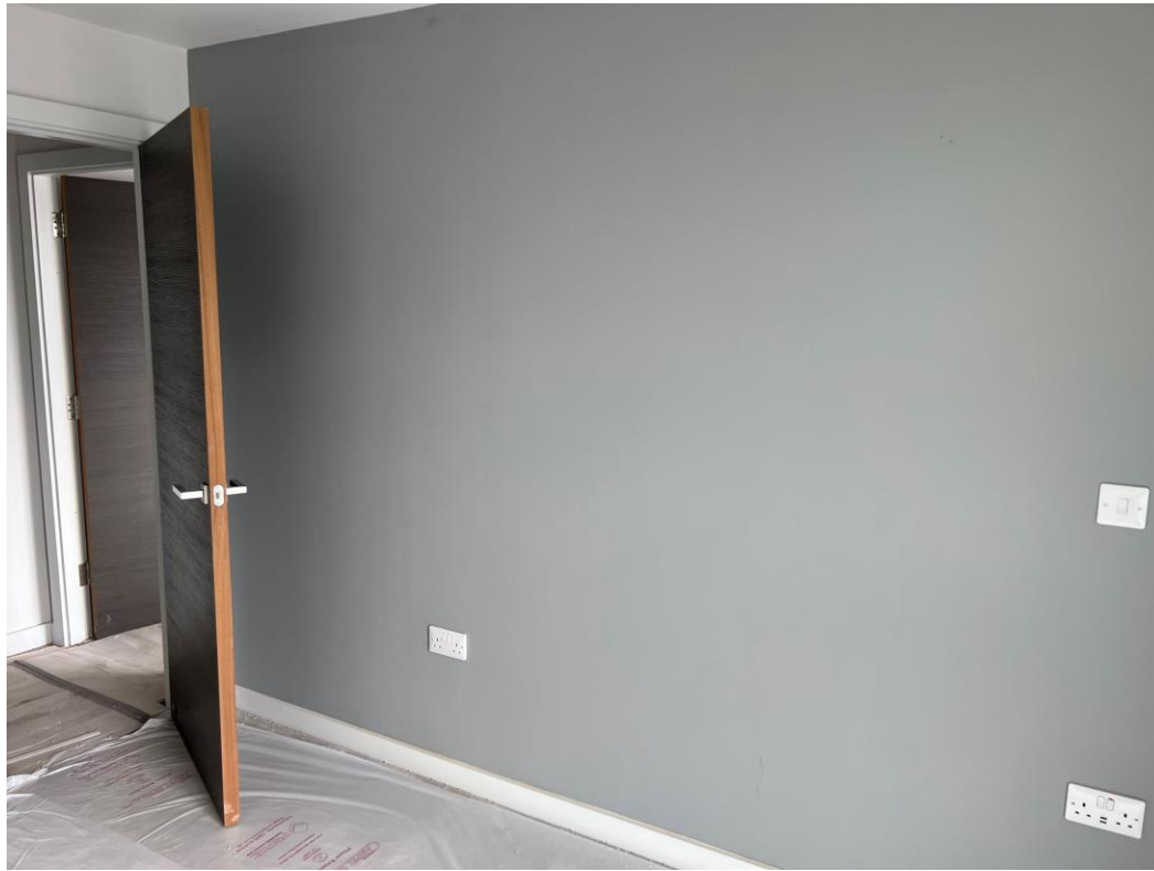
Level 1 – Internal doors installed
