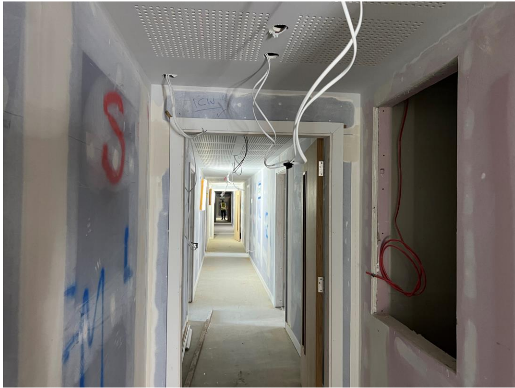
Level 5 – acoustic perforated board to corridor ceiling & fire doors
