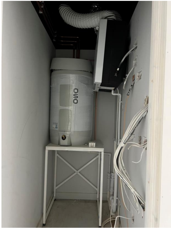
Level 3 – 2 nd fix mechanical & electrical
