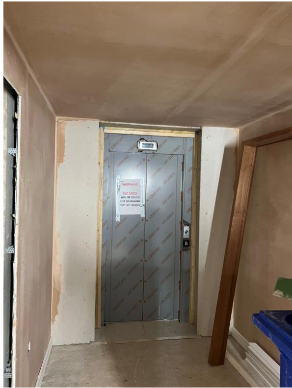
Level 5 – Lift lobby plastered
