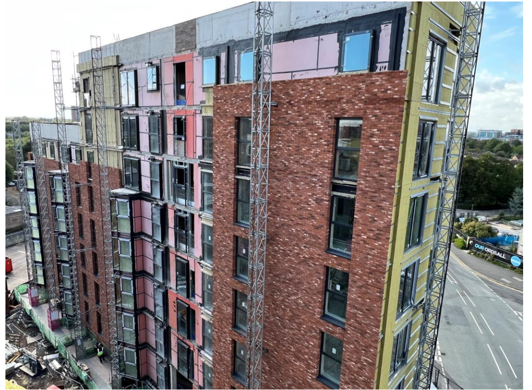
Block A wall insulation and brickwork
