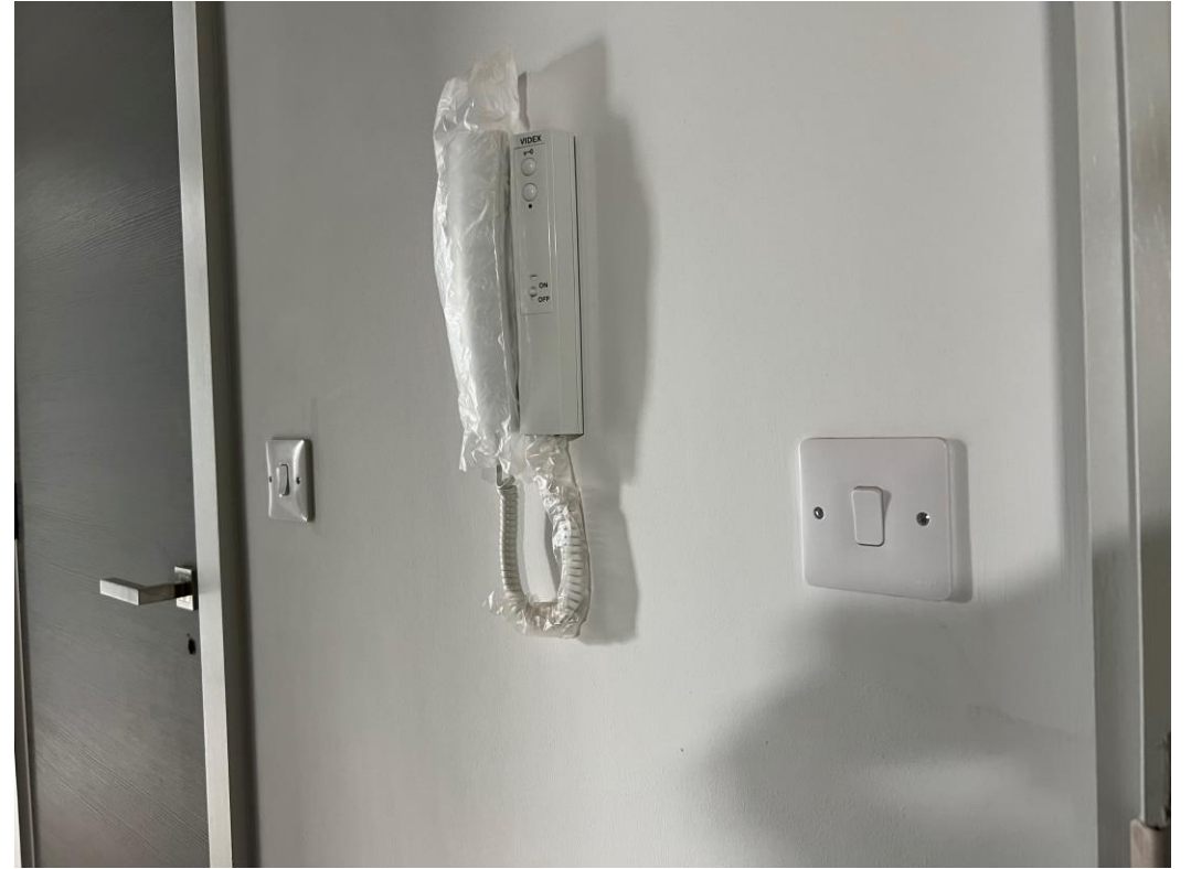
Level 2 – Internal doors installed
