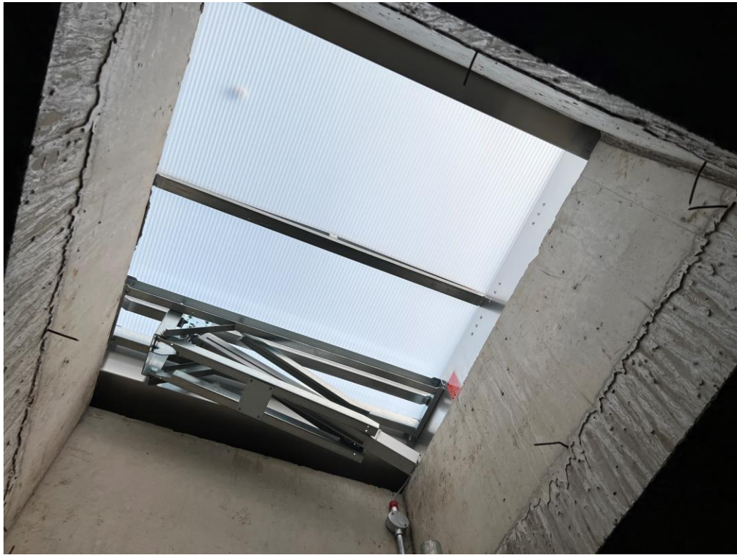
Level 6 – smoke vent installed
