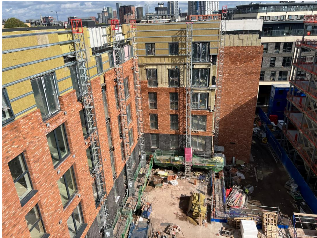
Block B wall insulation and cladding rail
