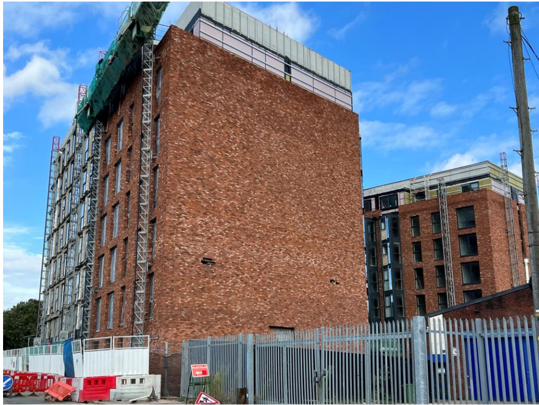
Worrall Street site view
