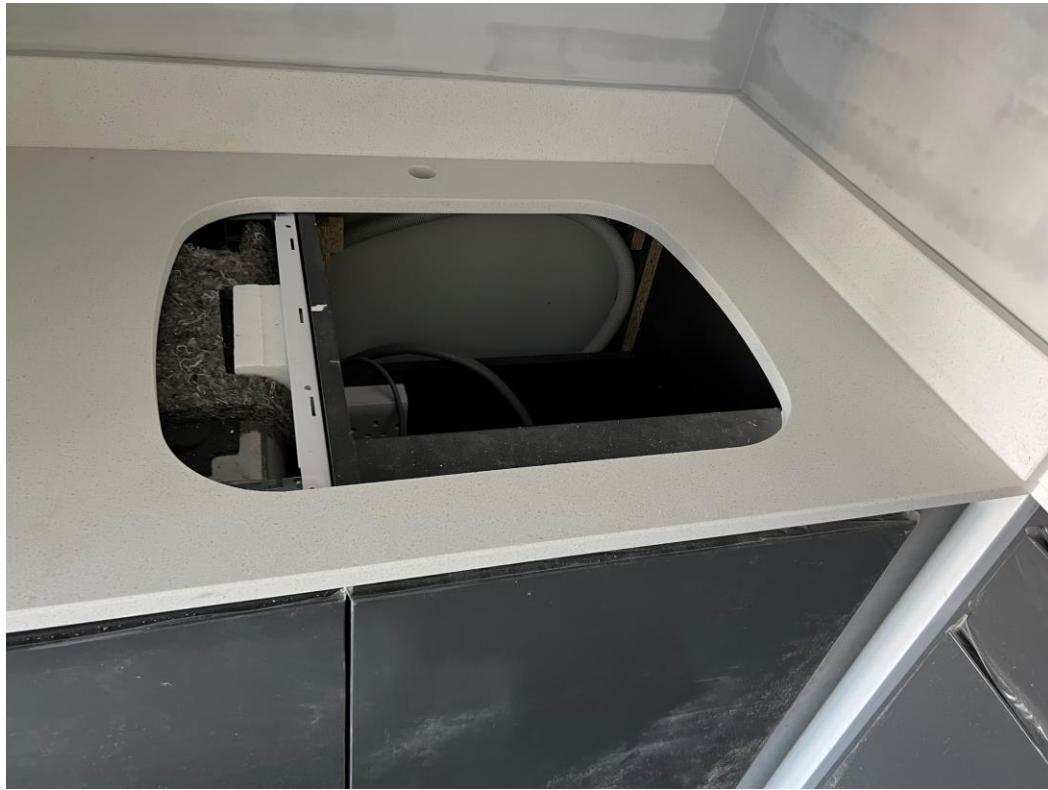
Level 5 – Kitchen worktop installed
