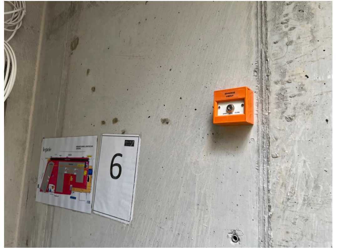
Level 6 – smoke vent control
