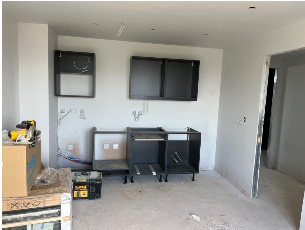
Level 8 – Kitchen units installed
