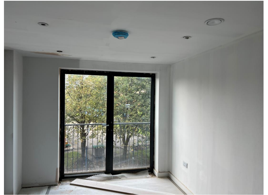
Level 2 – doorframes, skirting and architraves commenced
