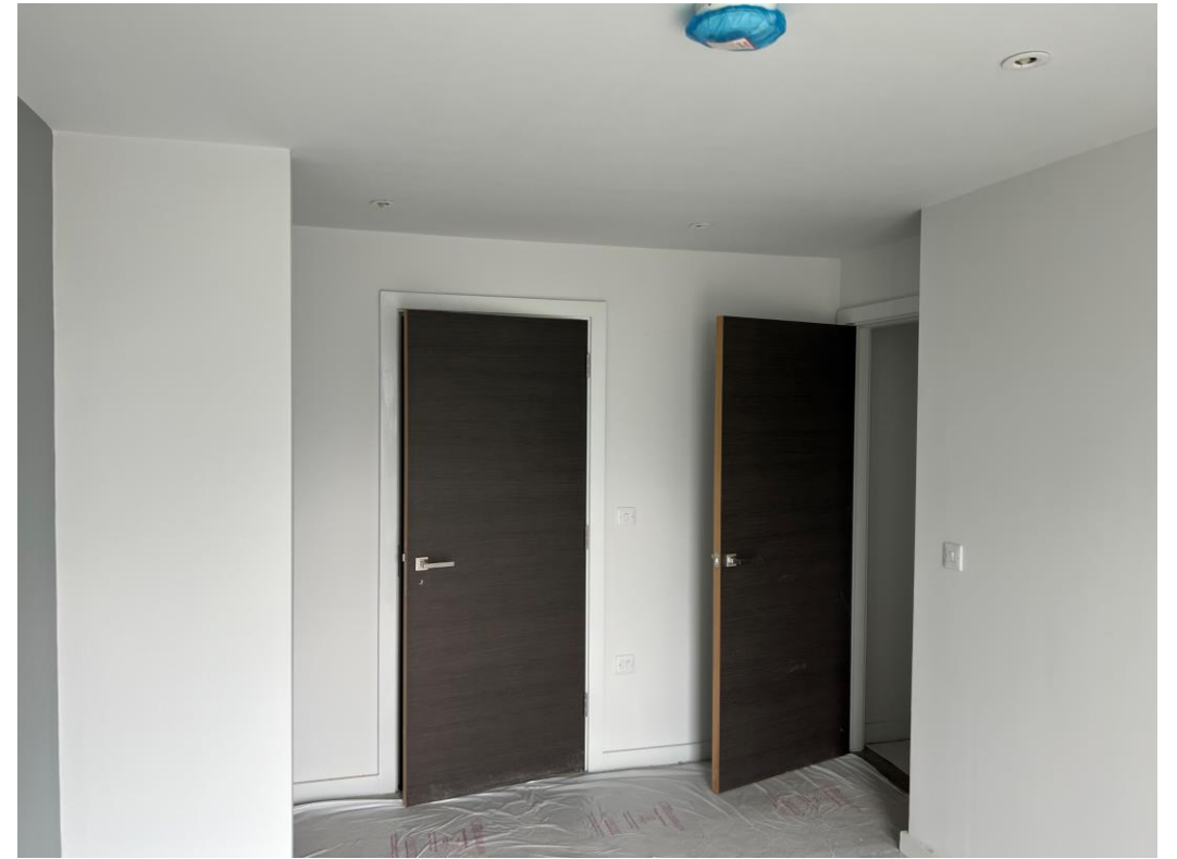
Level 1 – Internal doors installed
