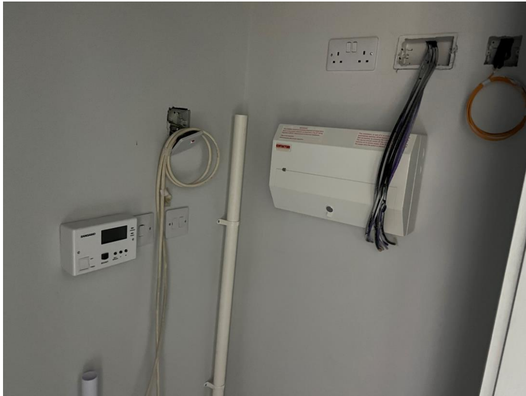
Level 6 – 2 nd fix electrical
