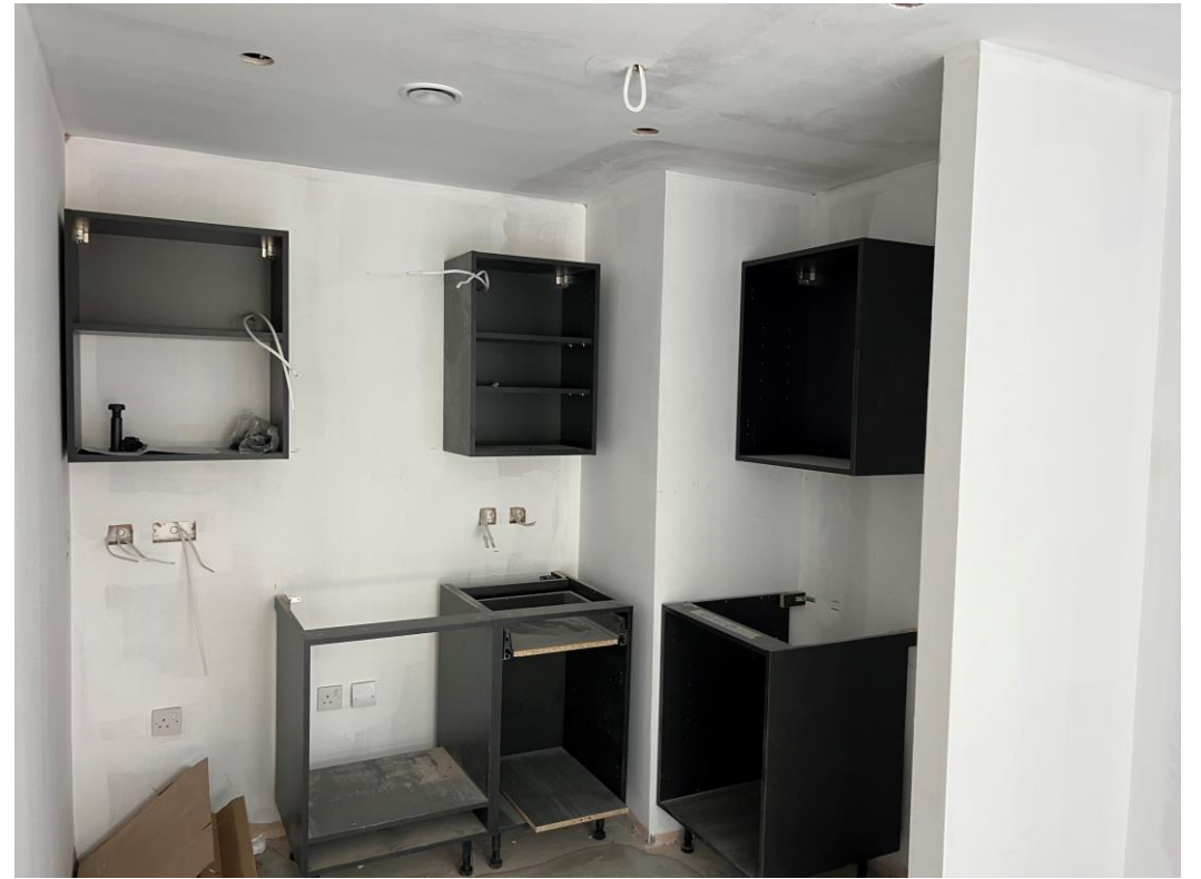
Level 1 – Kitchen units commenced
