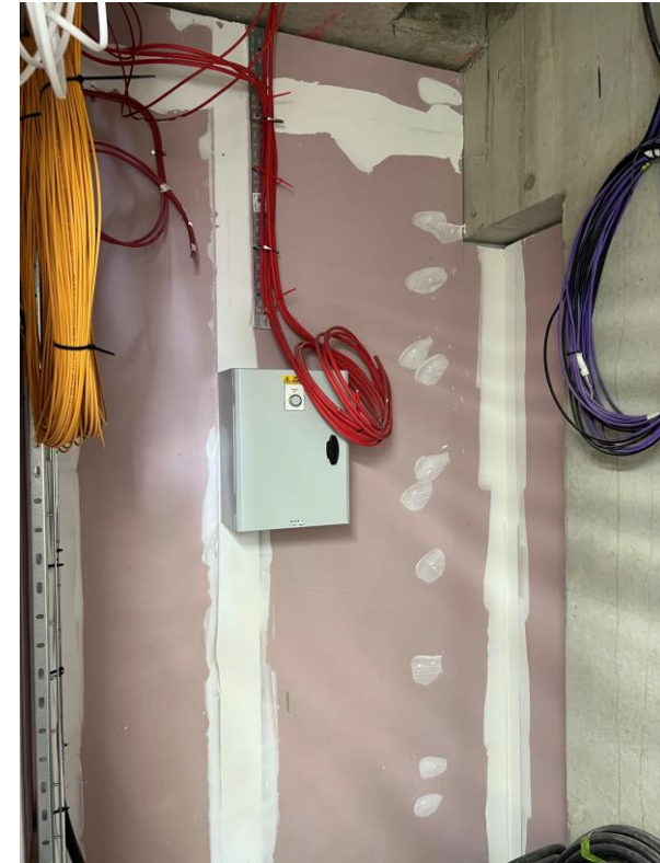
Level 7 – 2 nd fix electrical
