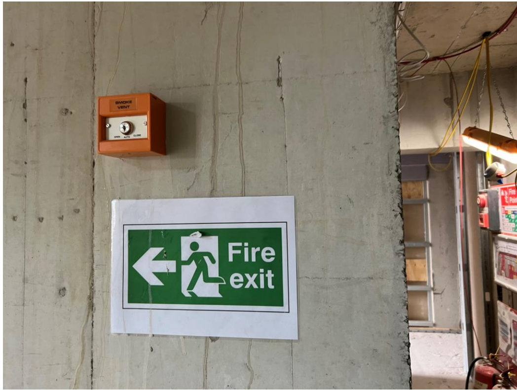
Level 7 – Smoke vent control
