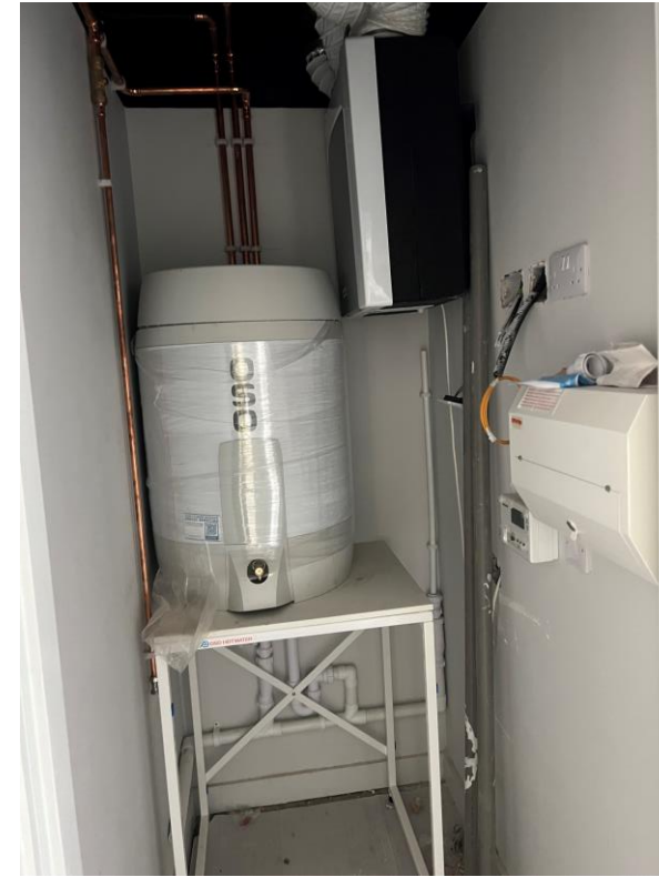
Level 5 – 2 nd fix mechanical
