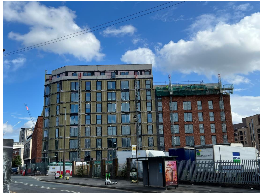
Ordsall Lane site view
