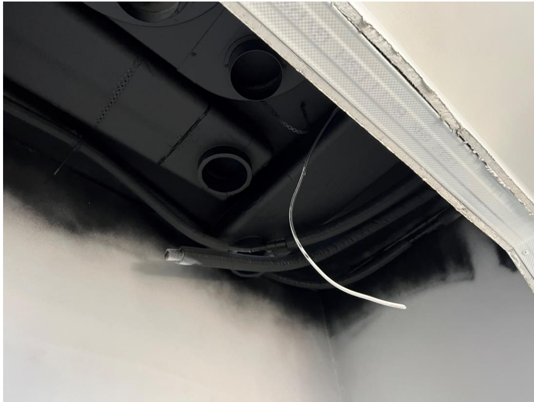
Level 8 – 1 st fix mechanical installation
