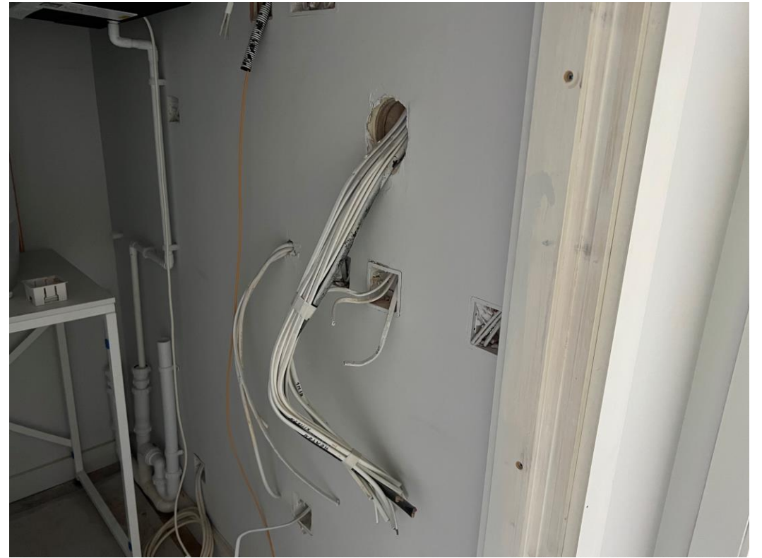
Level 3 – 2 nd fix mechanical & electrical
