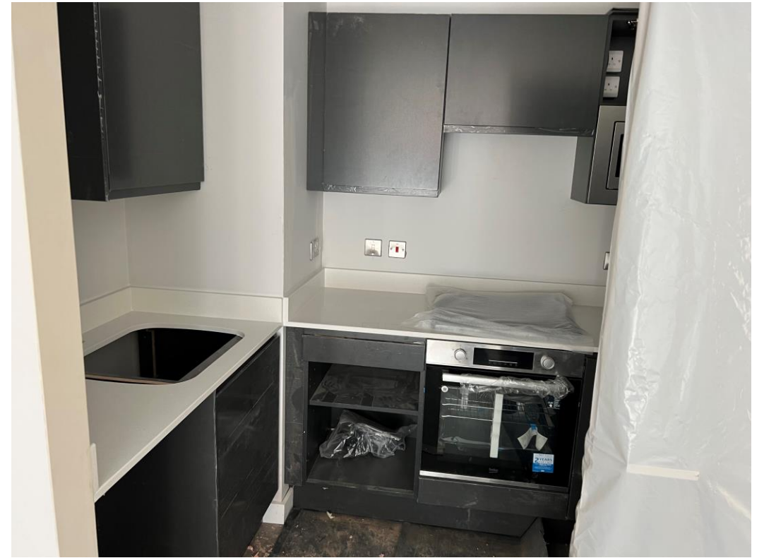
Level 5 – Kitchen units installed
