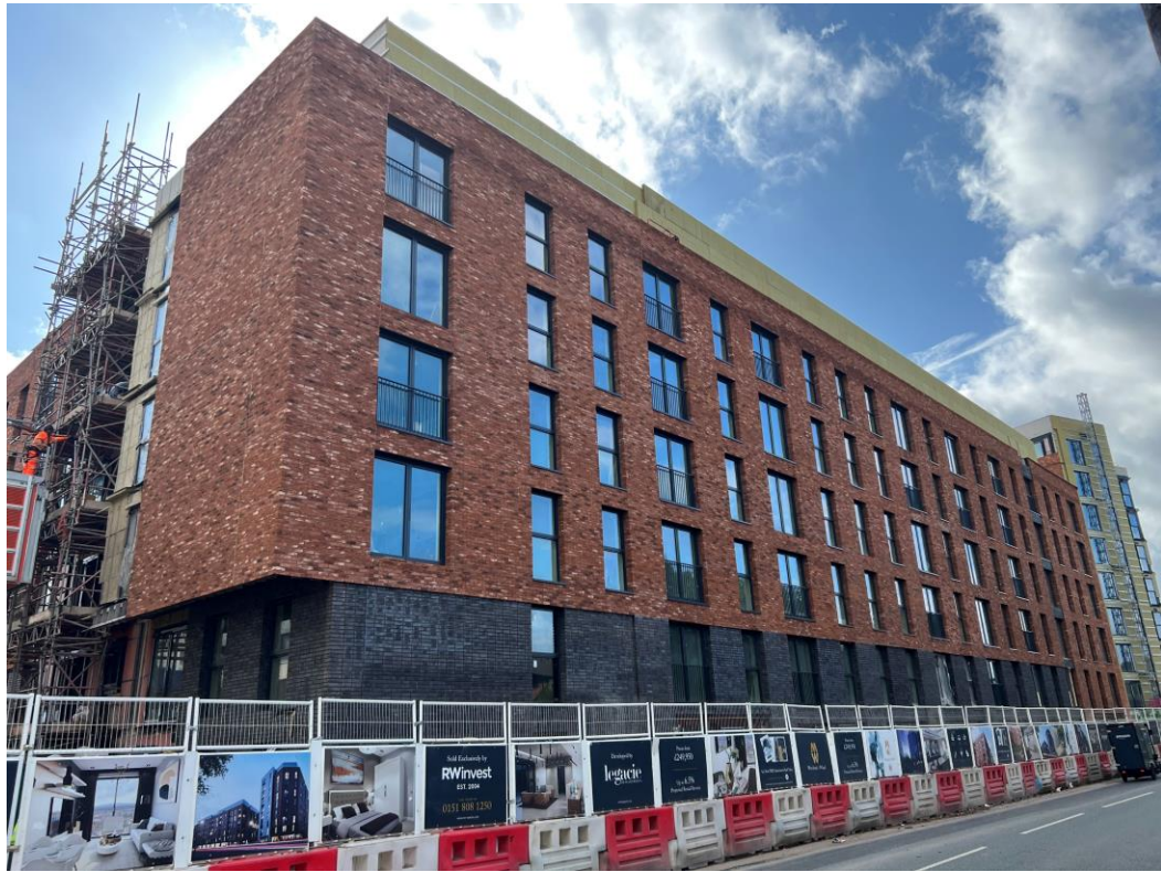
Ordsall Lane site view
