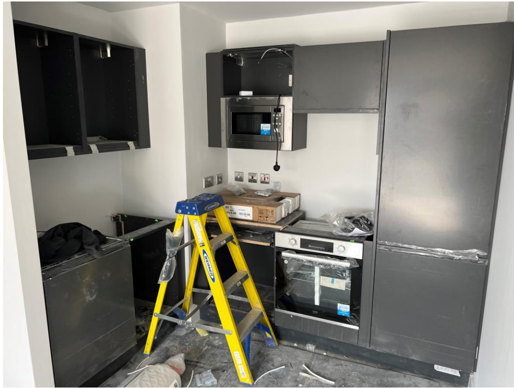
Level 5 – Kitchen units installed
