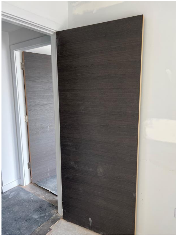
Level 2 – Internal doors installed
