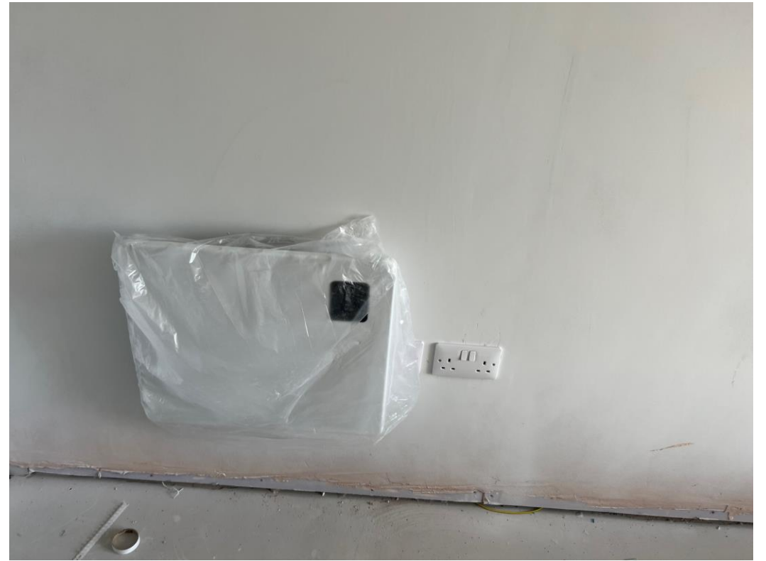
Level 7 – 2 nd fix wall heater installation
