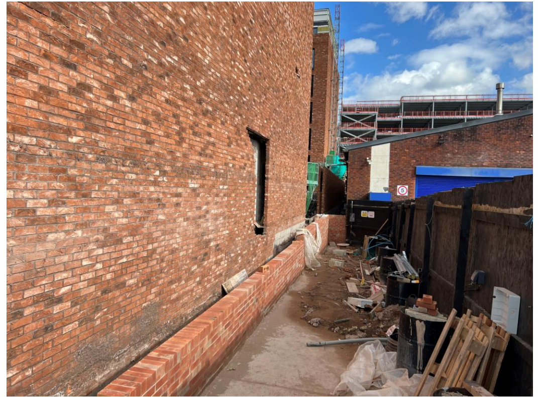
Worrall Street site view
