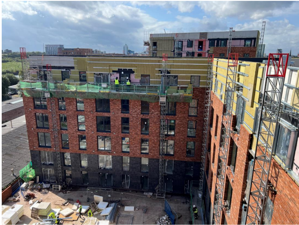
Block B wall insulation and cladding rail
