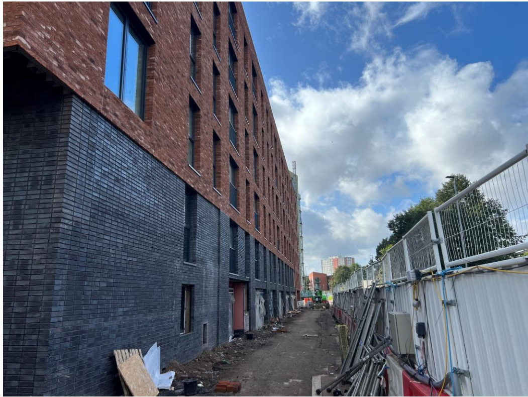
Ordsall Lane site view
