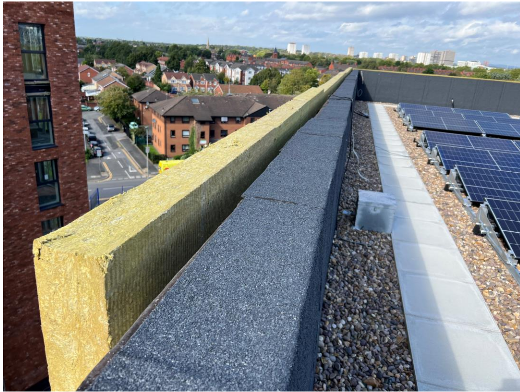
Block B Insulation detail prior to capping parapet
