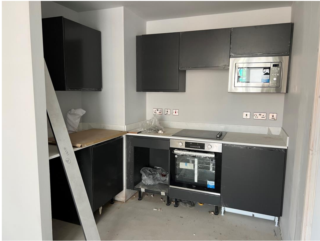
Level 5 – Kitchen units worktop & appliances installed
