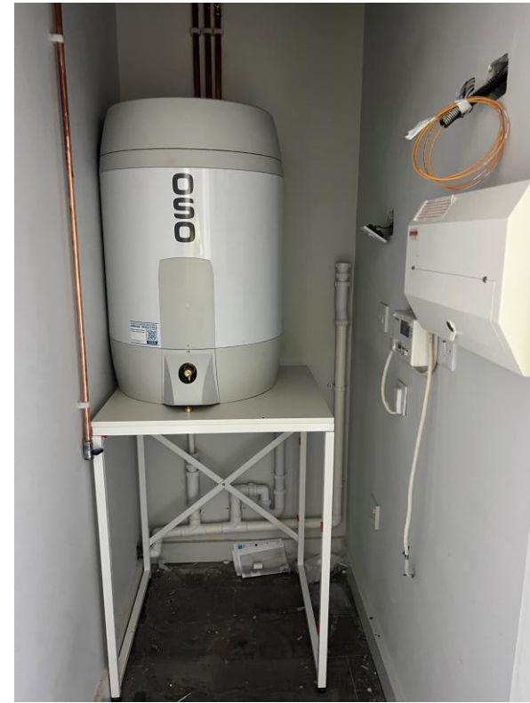
Level 6 – 2 nd fix mechanical
