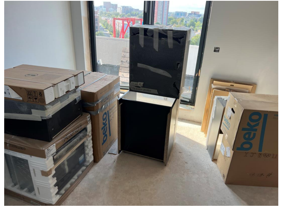
Level 8 – Kitchen units installed
