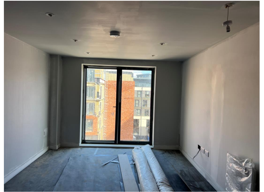
Level 5 – Decorations commenced walls and ceilings
