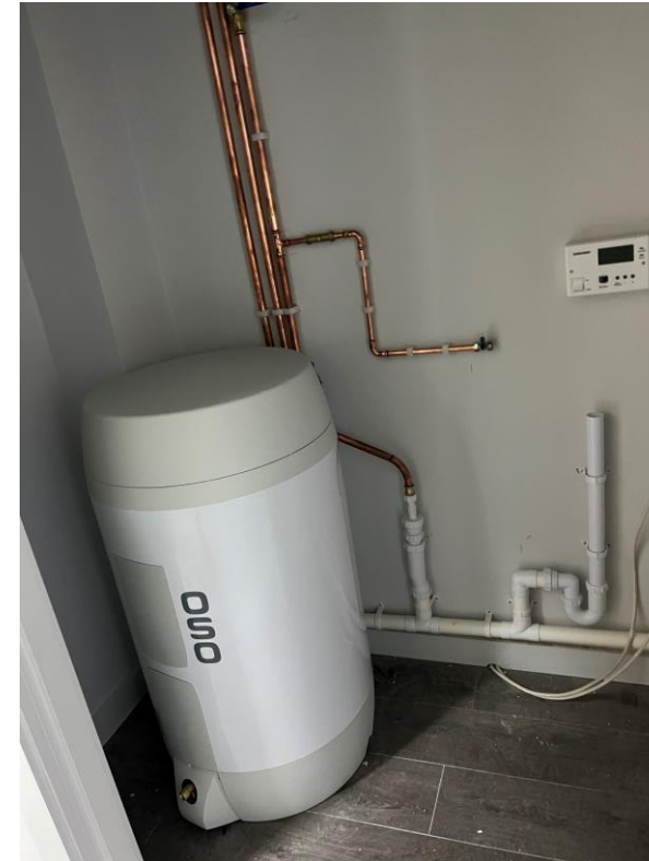
Level 6 – 2 nd fix mechanical
