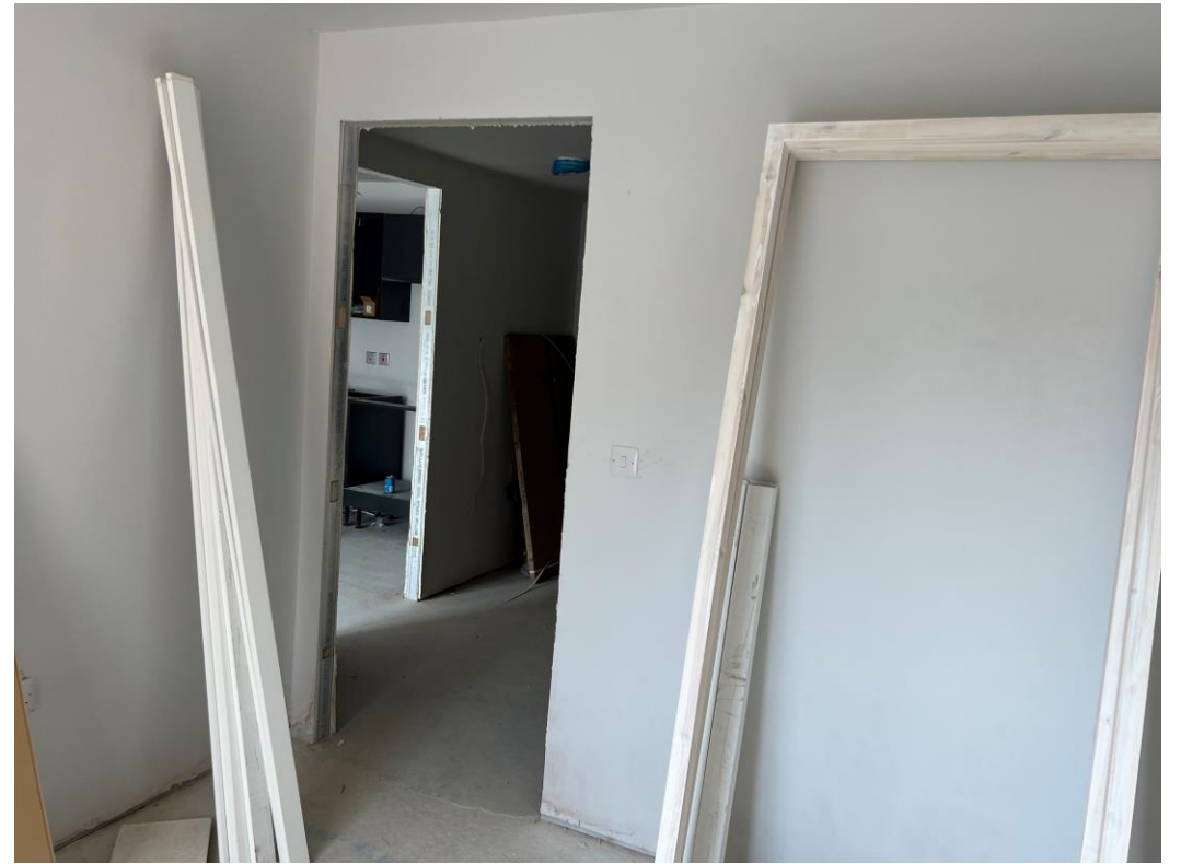
Level 4 – Doorframes & architrave being installed
