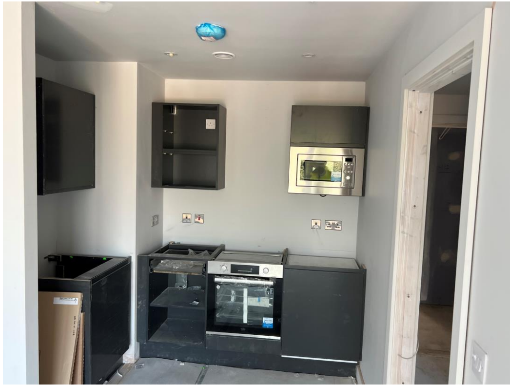
Level 4 – Kitchen units installed
