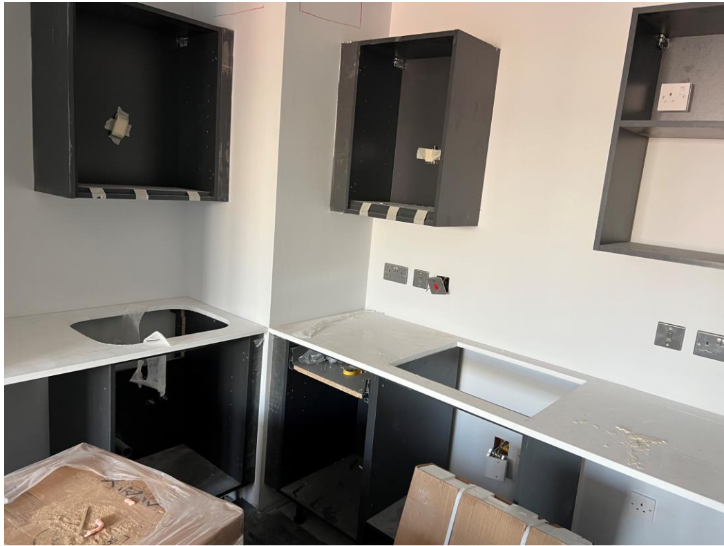
Level 6 – Kitchen units worktop installed
