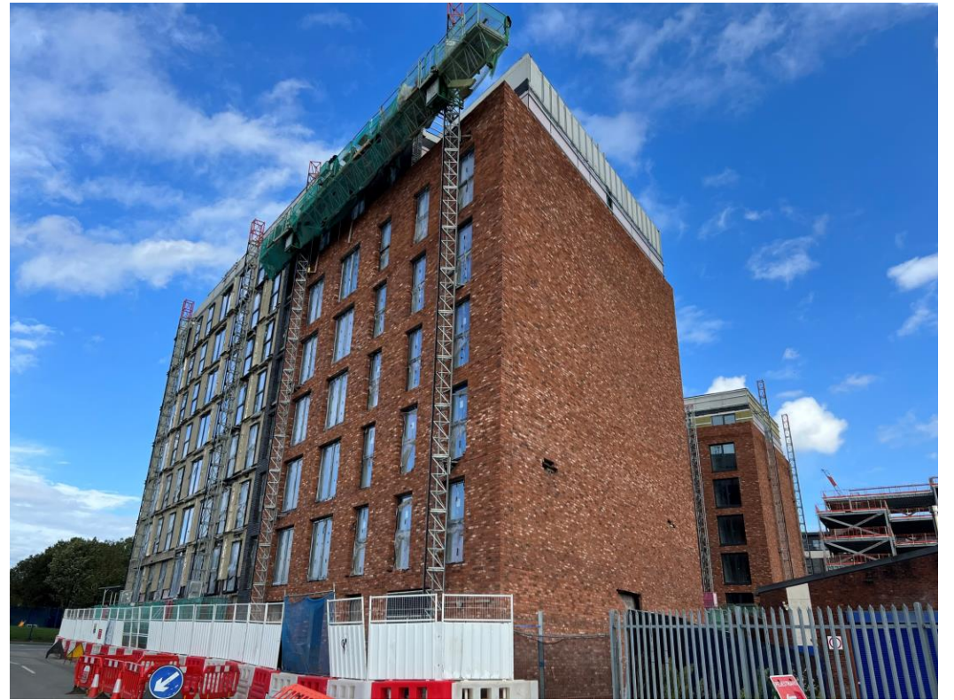
Worrall Street site view
