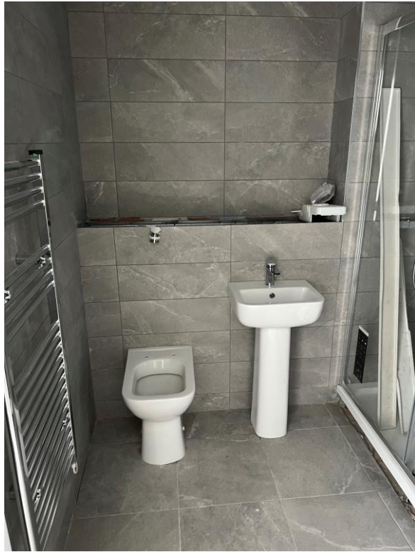
Level 6 – Sanitary appliances installed
