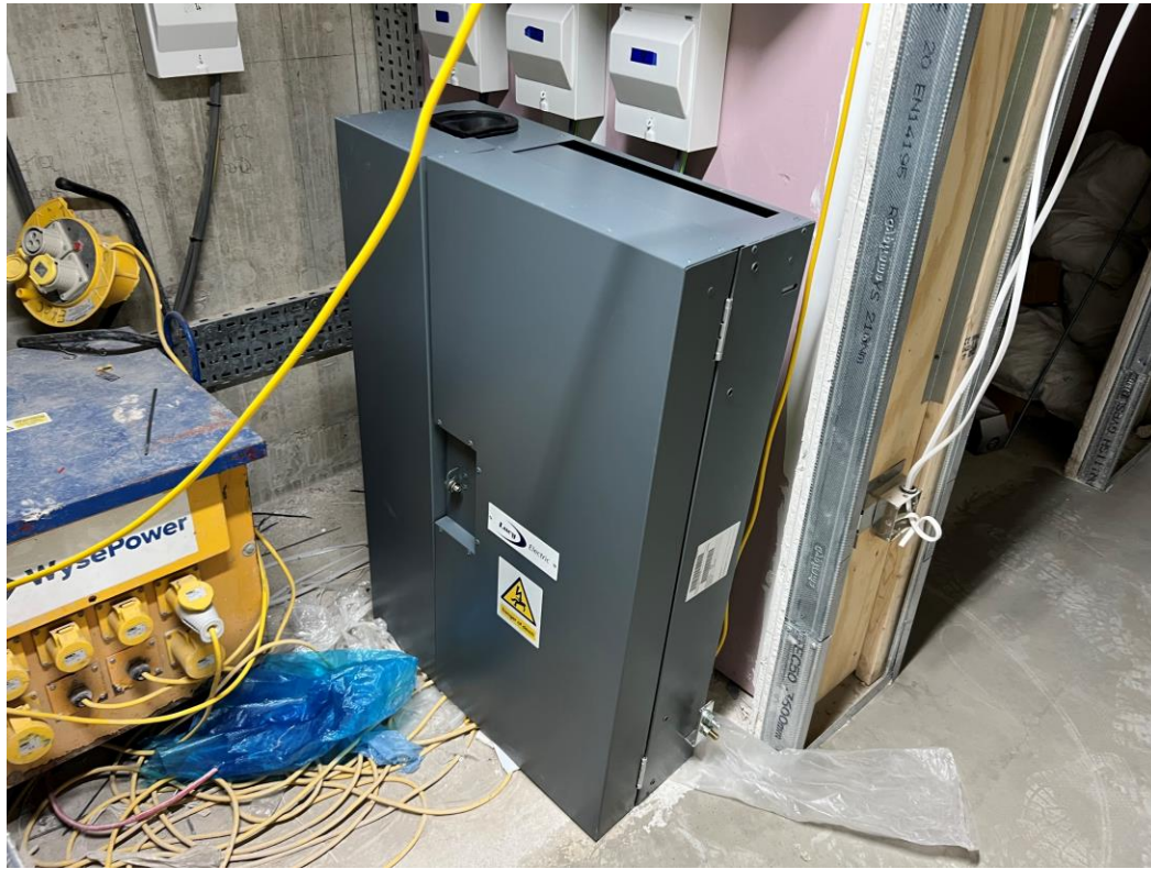
Level 6 – 2 nd fix electrical
