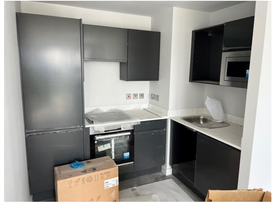
Level 4 – Kitchen complete
