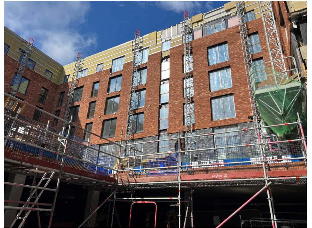
Block B wall insulation and cladding rail
