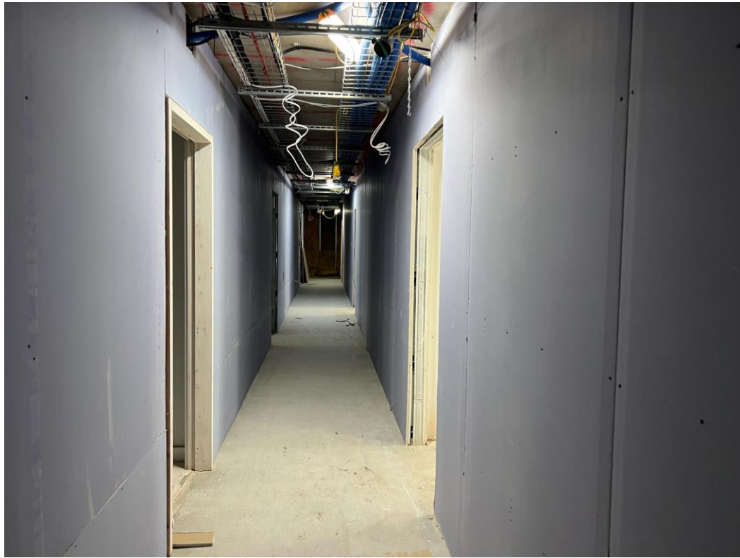
Level 1 – corridor walls boarded
