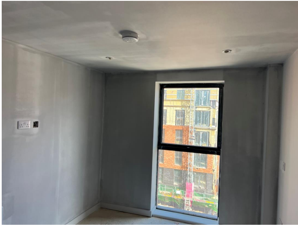
Level 5 – Decorations commenced walls and ceilings
