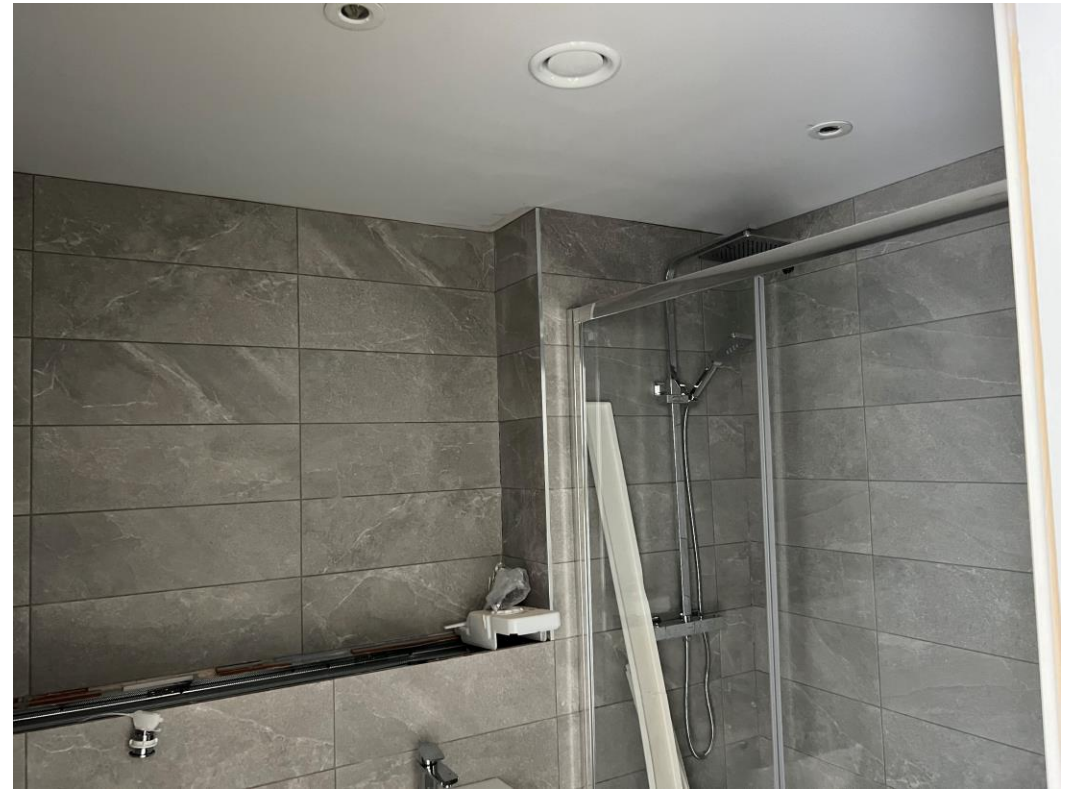
Level 6 – Sanitary appliances installed
