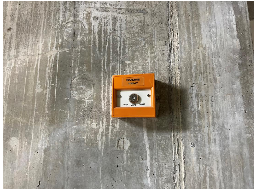
Level 6 – smoke vent control
