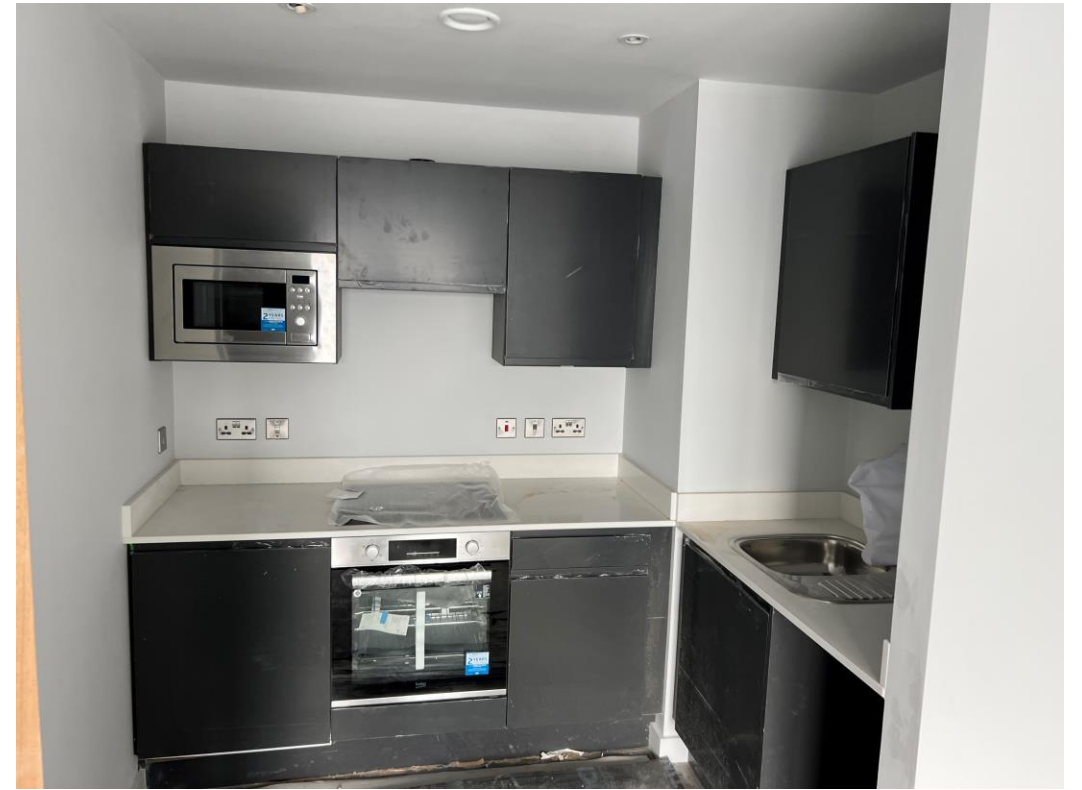
Level 6 – Kitchen units and appliances installed
