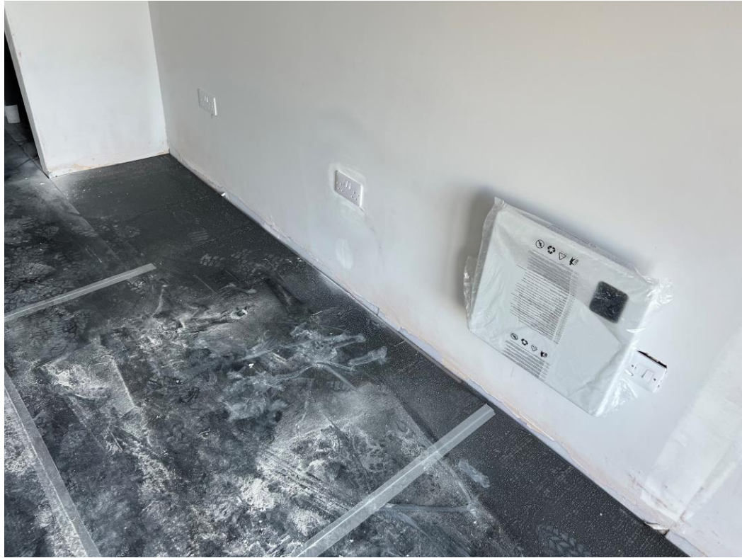
Level 5 – wood laminate flooring
