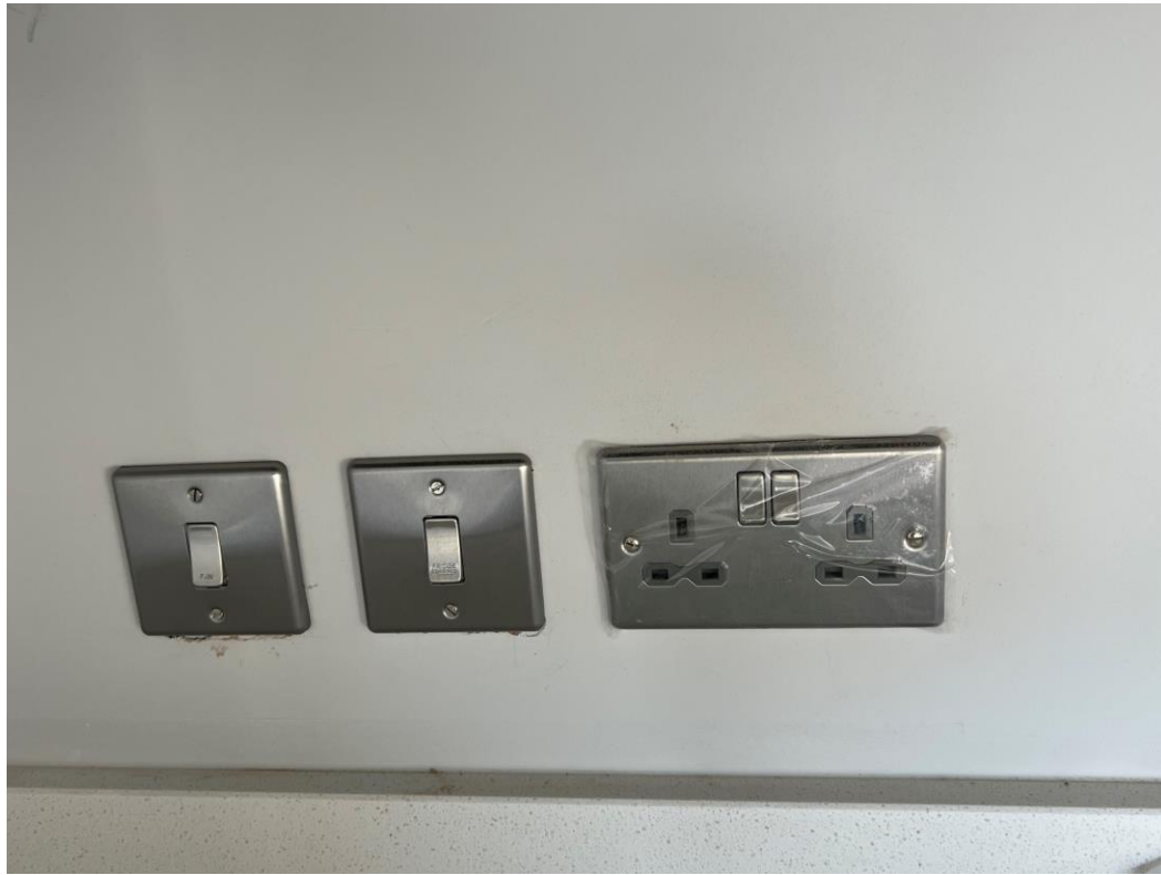
Level 6 – 2 nd fix electrical sockets
