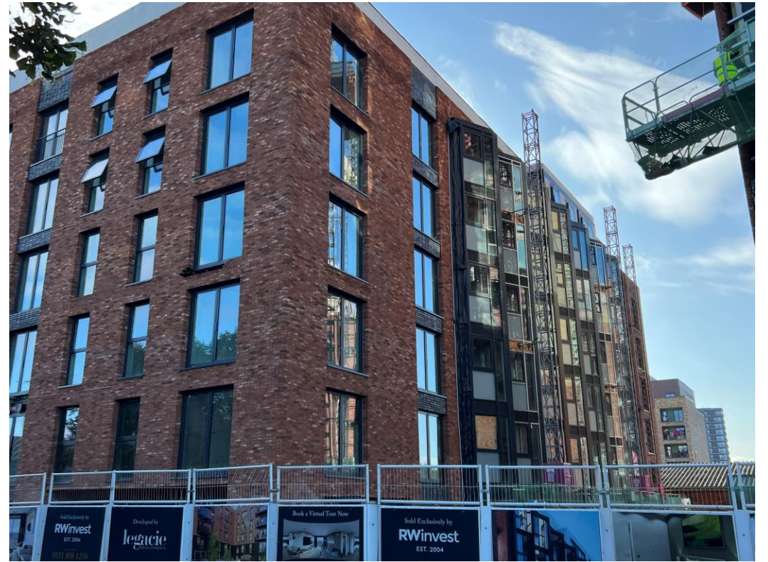
Ordsall Lane site view
