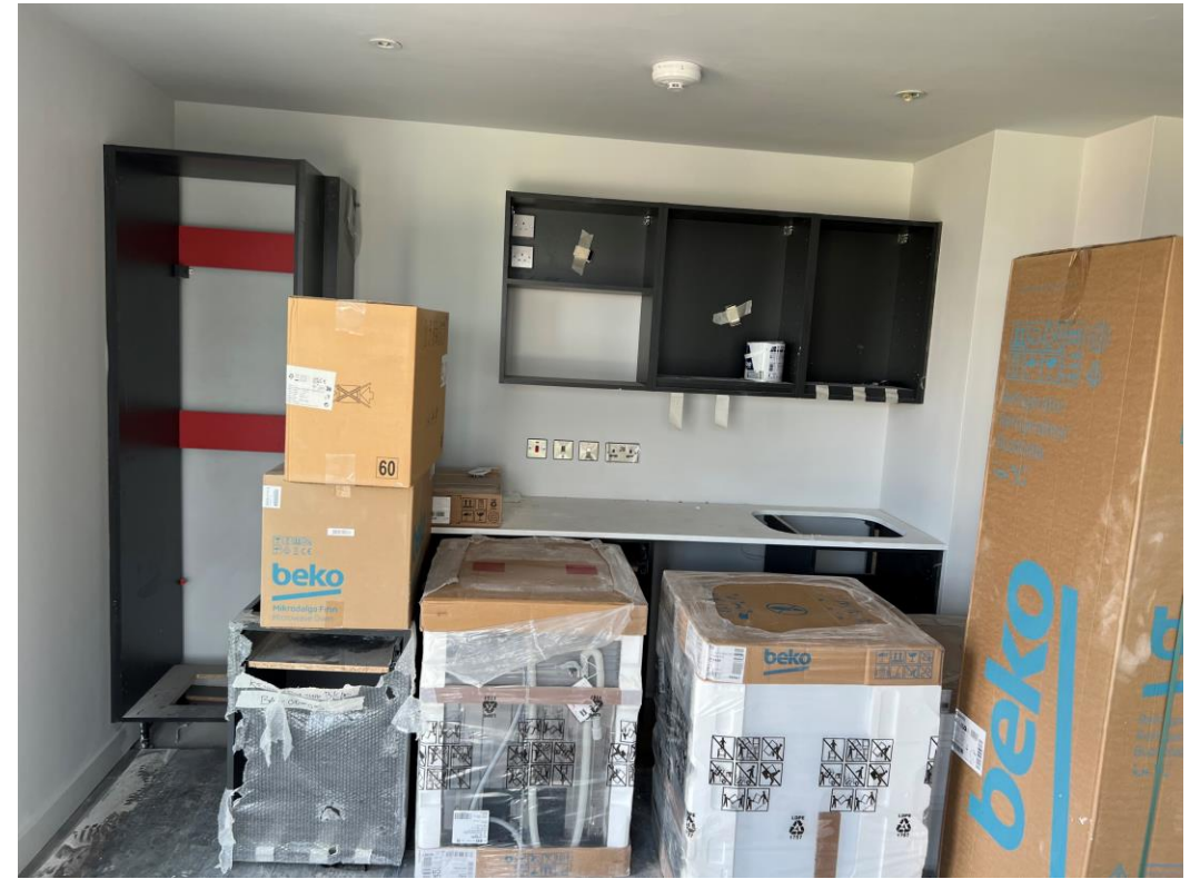
Level 6 – Kitchen units installed
