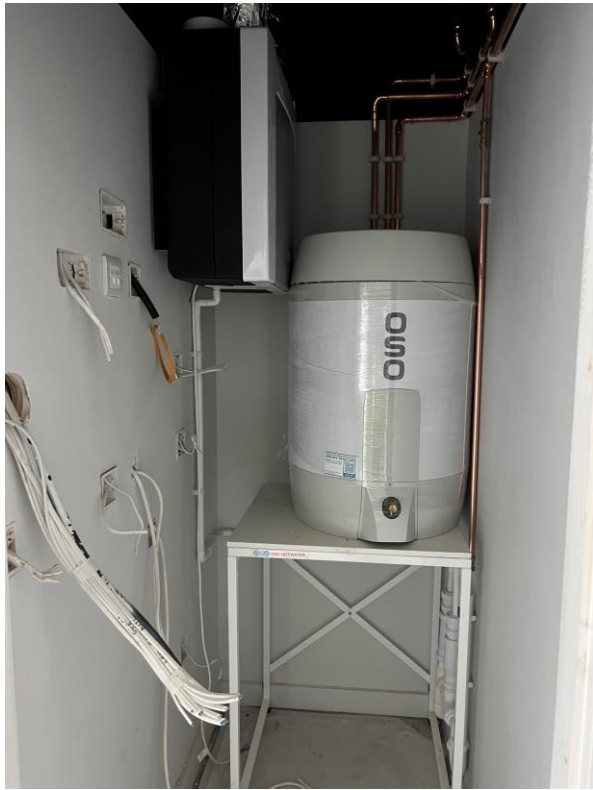
Level 3 – 2 nd fix mechanical
