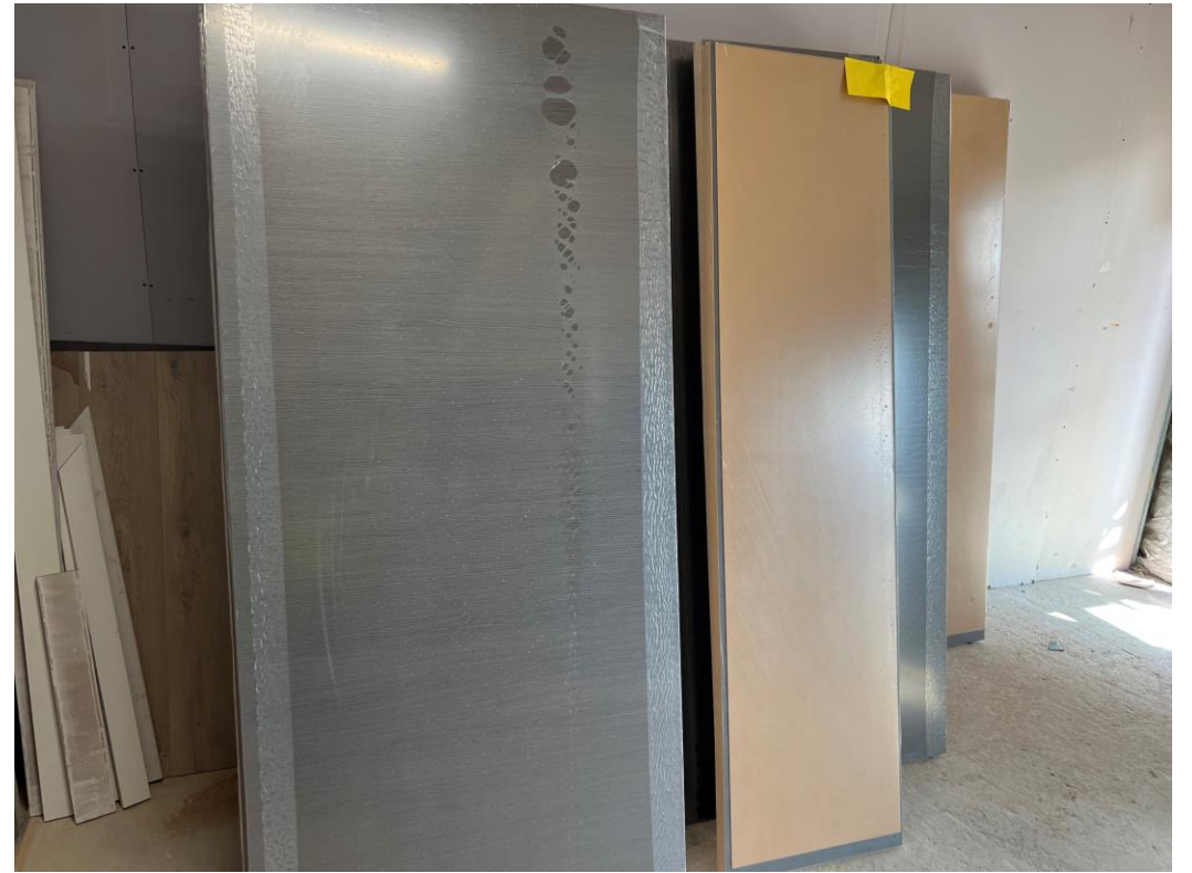
Level 2 – Internal woodgrain doors
