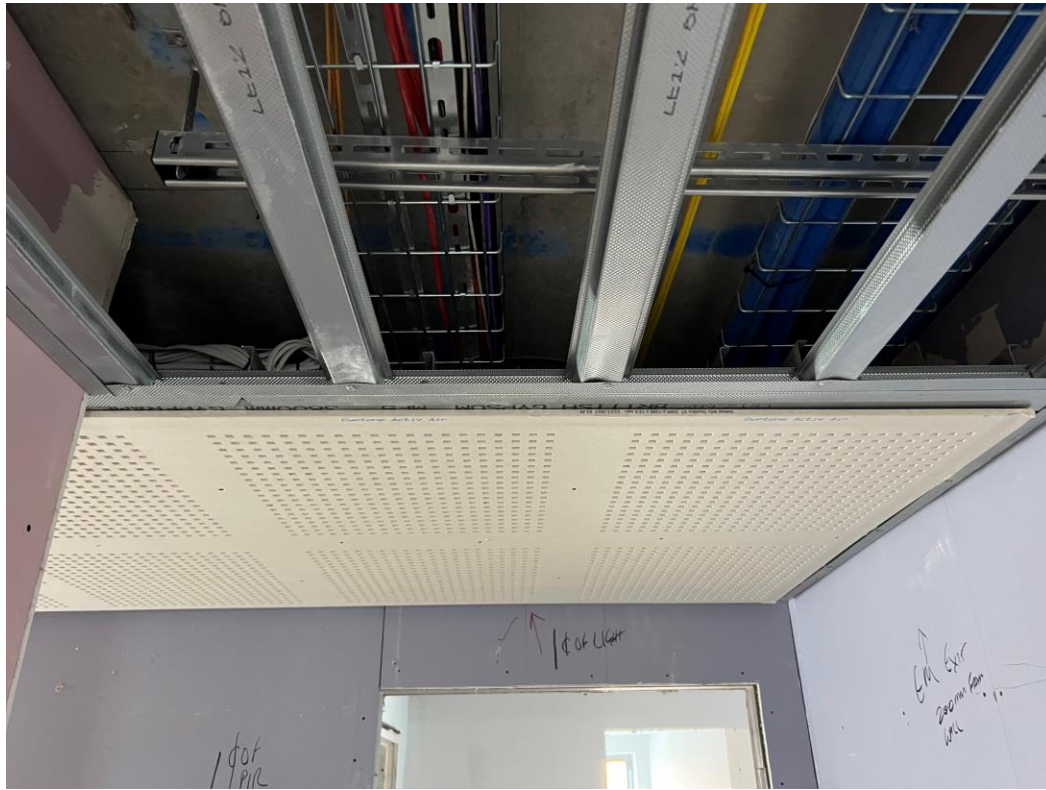
Level 5 – acoustic perforated board to corridor ceiling
