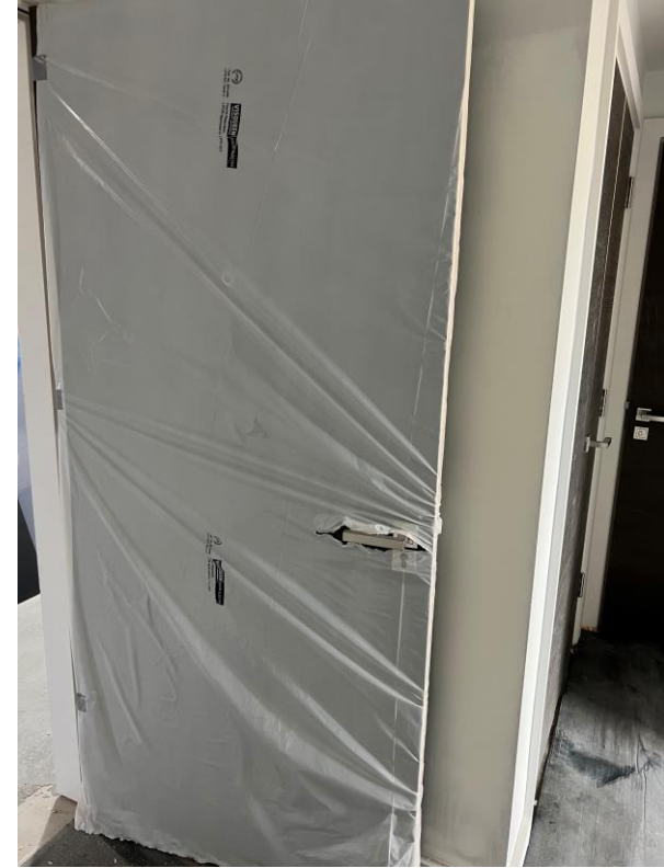
Level 6 – Internal woodgrain doors installed
