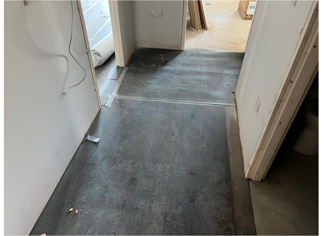
Level 5 – wood laminate flooring
