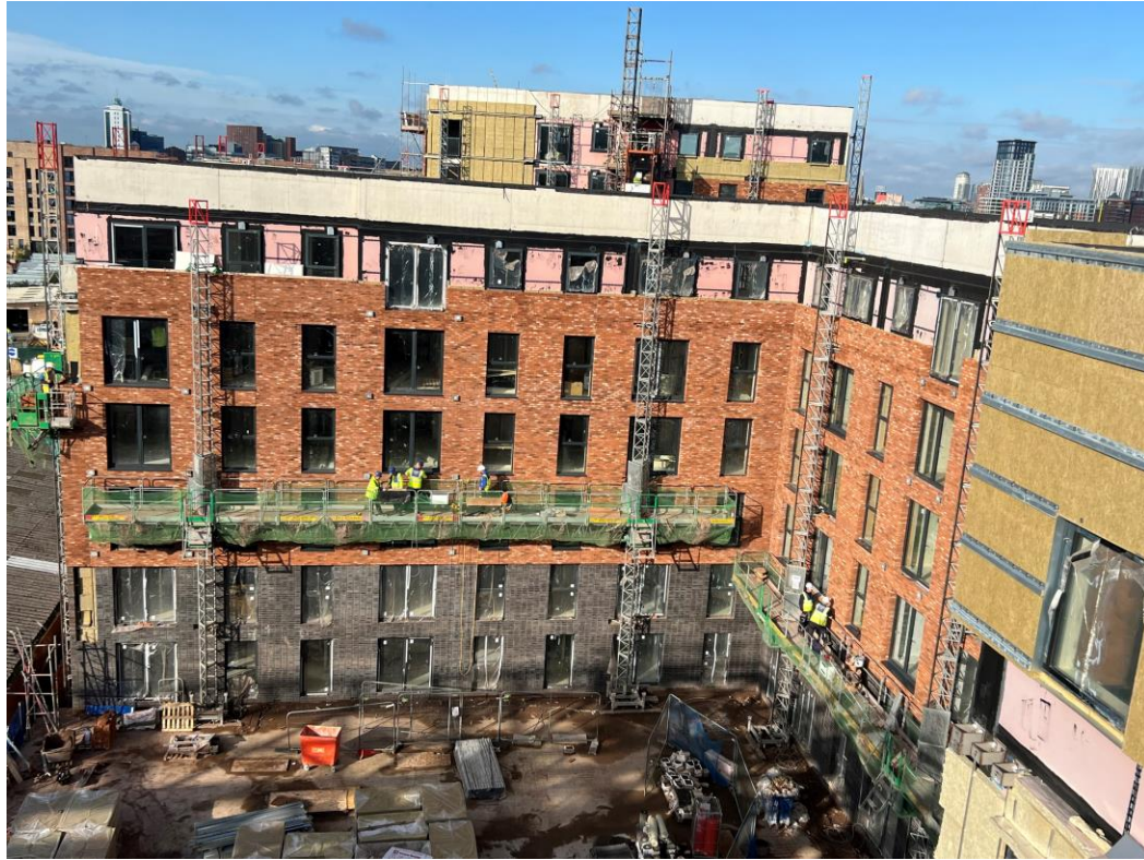
Block B wall insulation and brickwork
