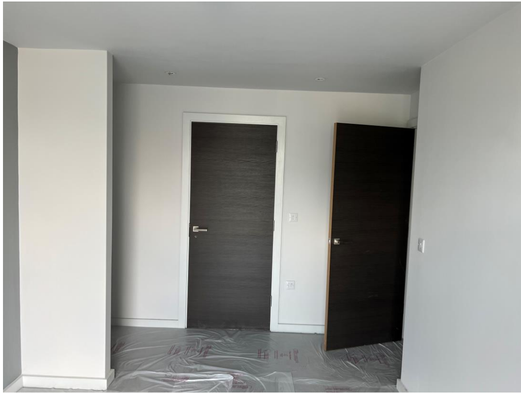
Level 1 – Internal woodgrain doors installed
