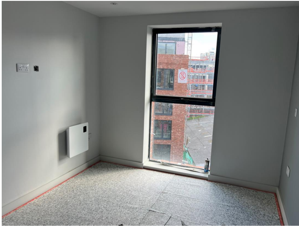
Level 5 – carpet floor covering installation
