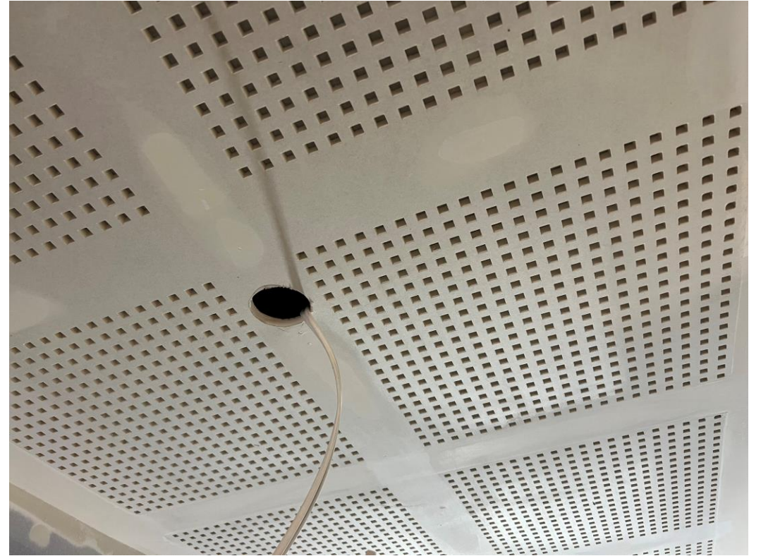
Level 6 – acoustic perforated board to corridor ceiling
