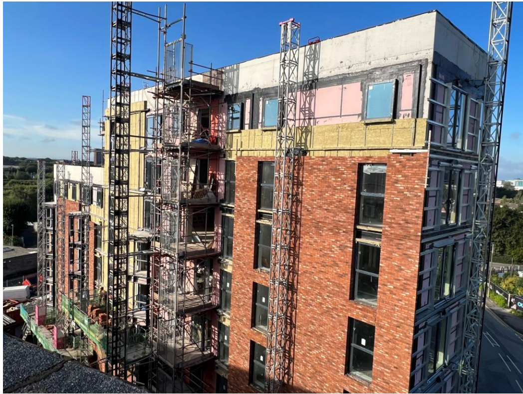
Block A wall insulation and brickwork
