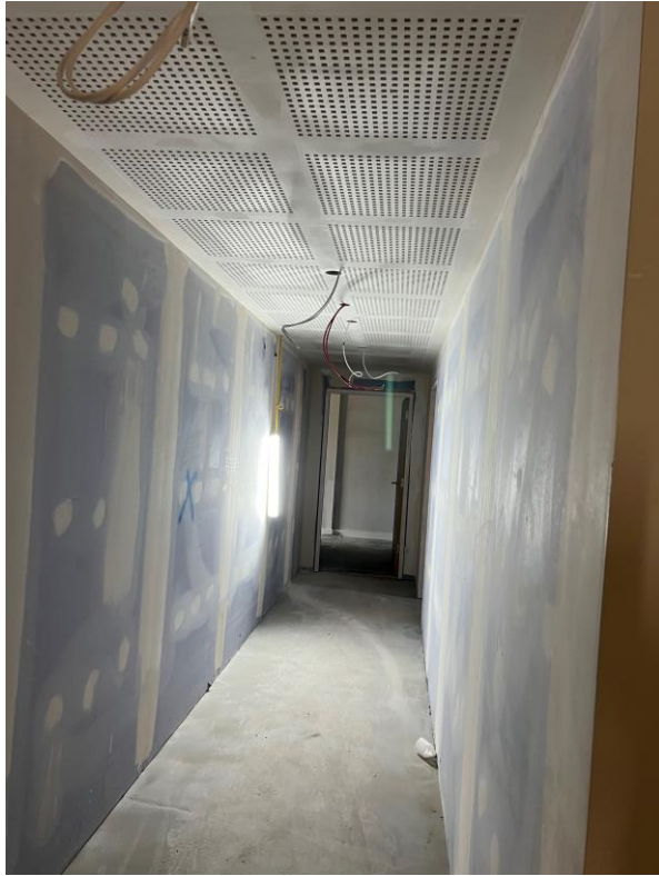
Level 6 – acoustic perforated board to corridor ceiling
