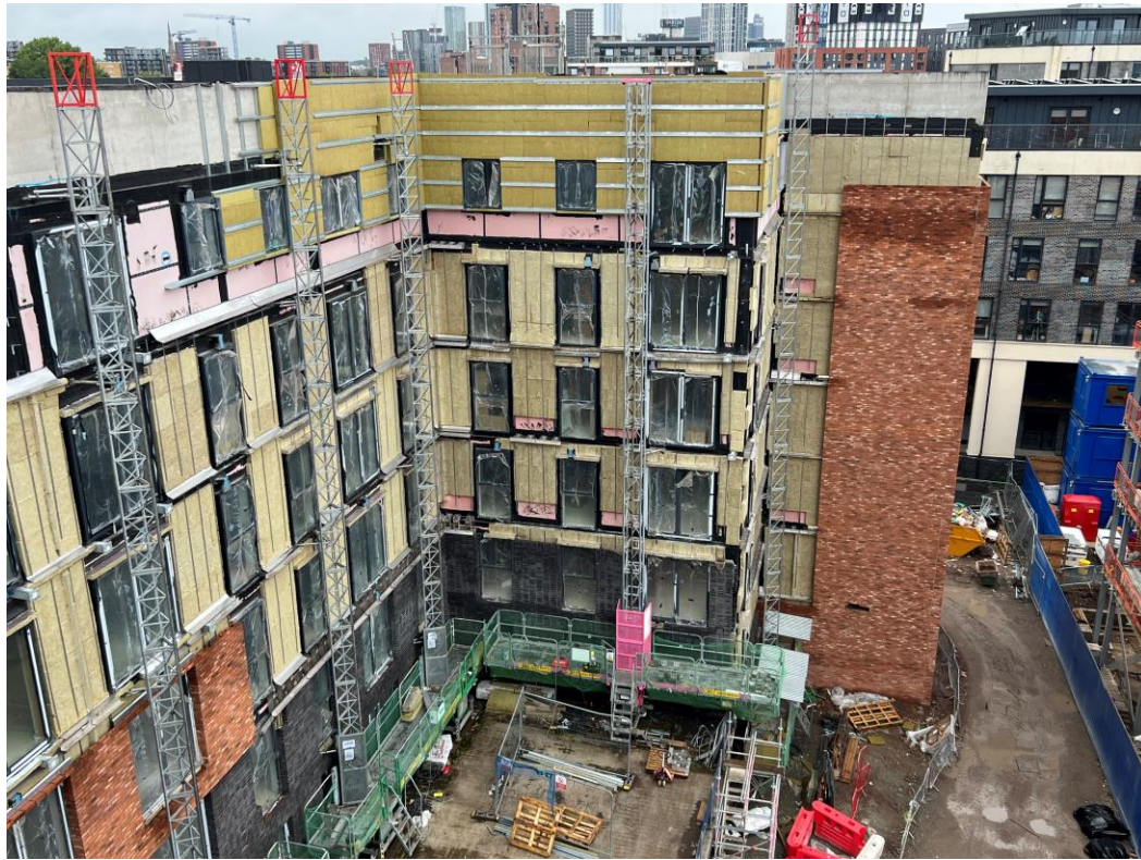
Block B cladding rail and insulation
