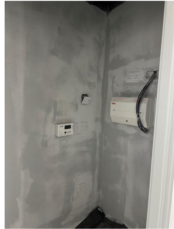
Level 6 – 2 nd fix electrical
