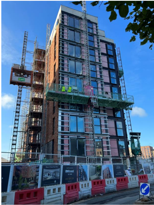
Ordsall Lane site view
