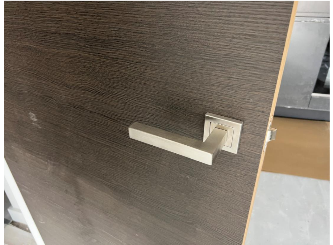
Level 1 – Internal woodgrain doors
