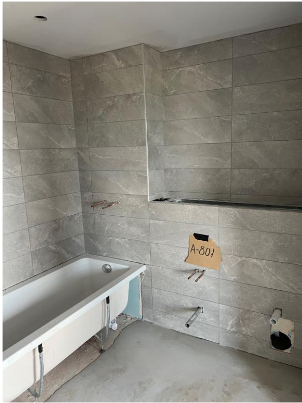
Level 8 – wall and floor tiling
