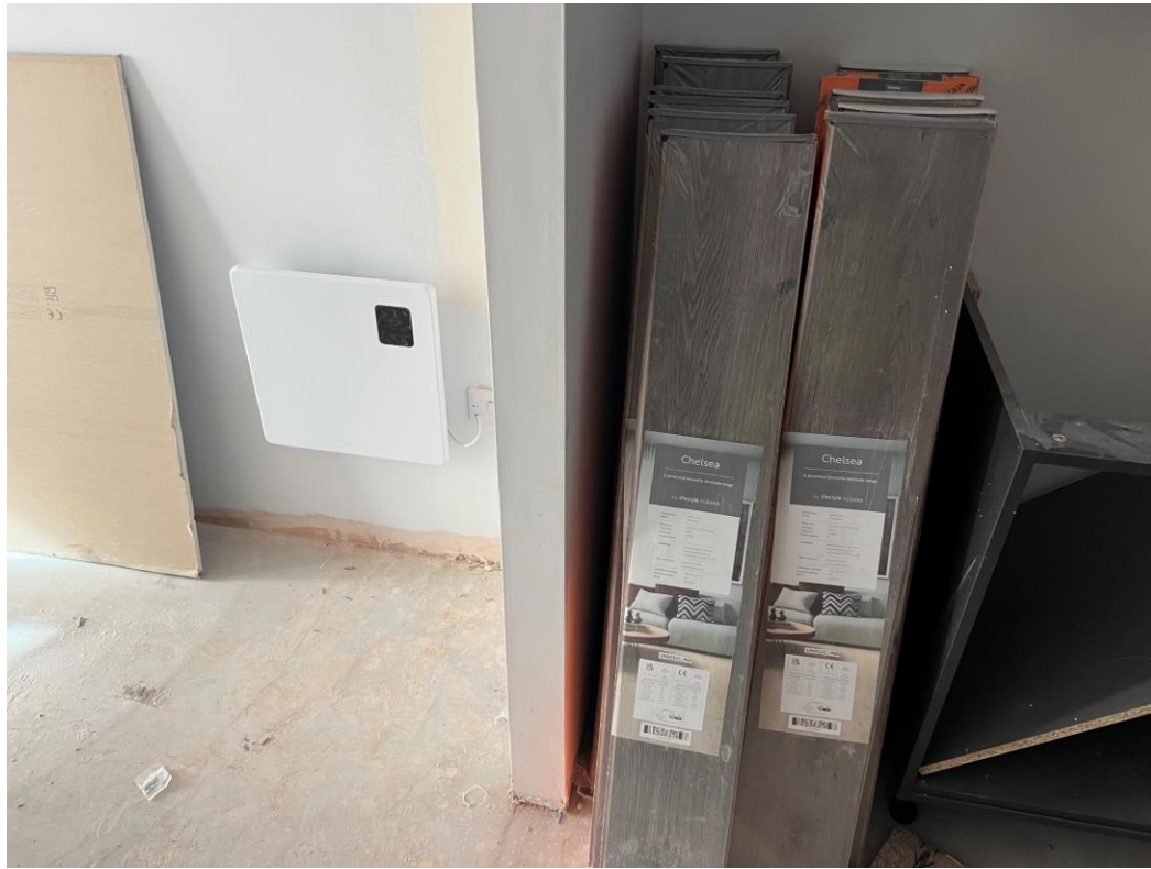
Level 5 – wood laminate flooring
