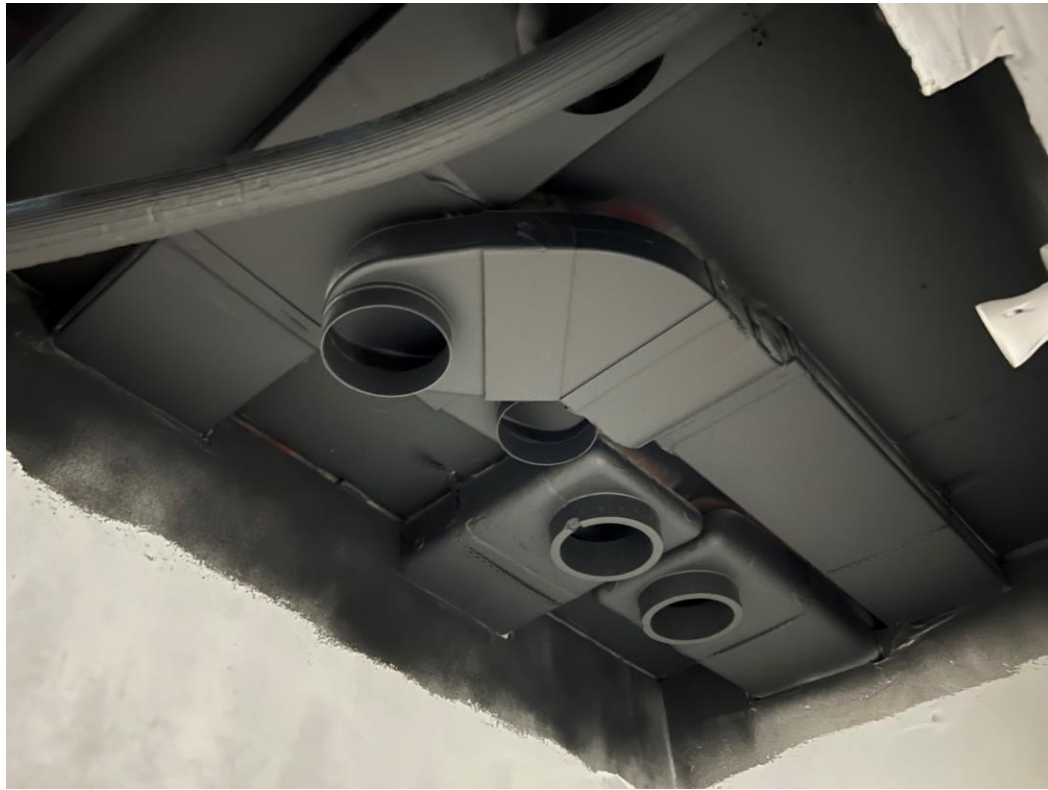
Level 6 – 2 nd fix mechanical installation
