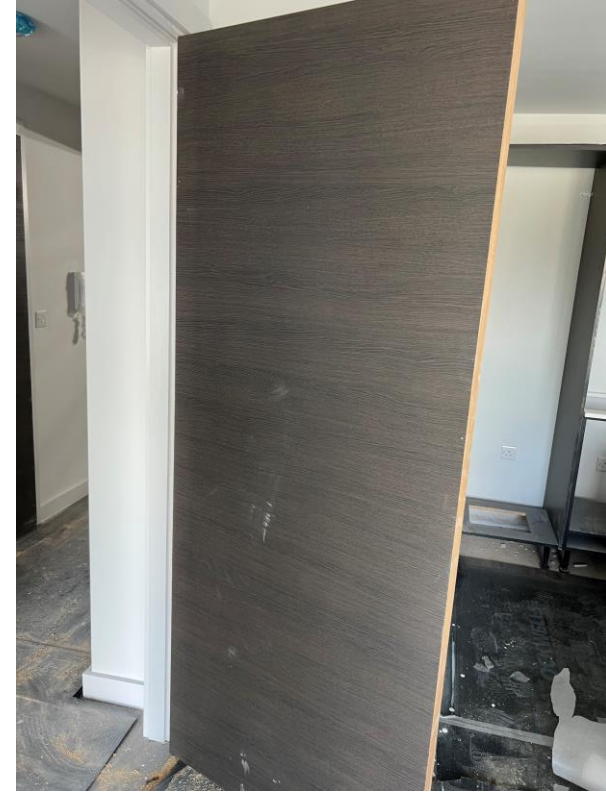
Level 2 – Internal woodgrain doors installed
