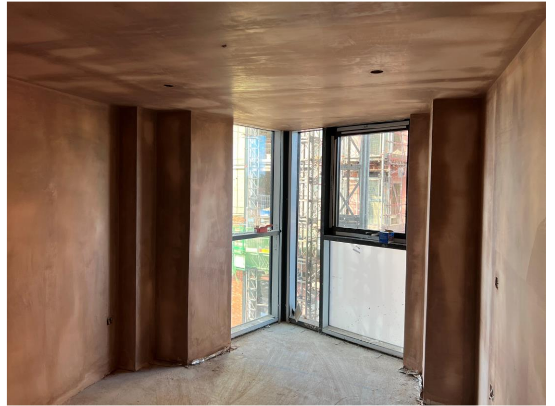
Level 5 – walls and ceiling plaster skim finish
