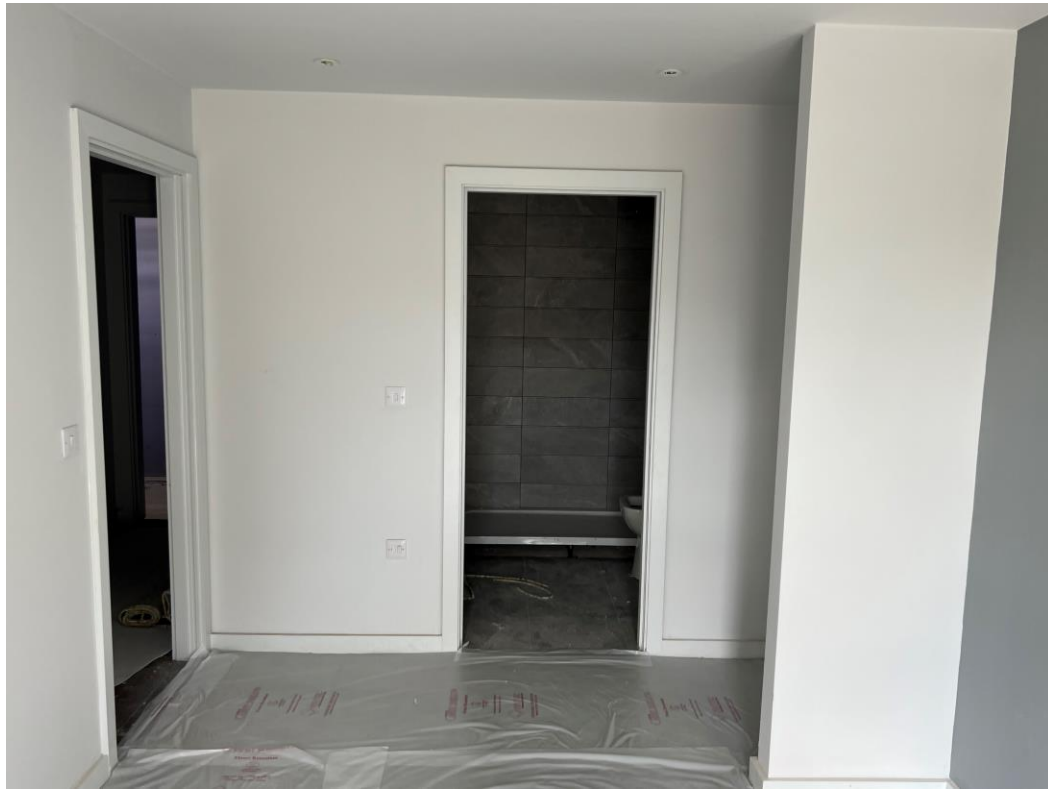
Level 4 – carpet floor covering
