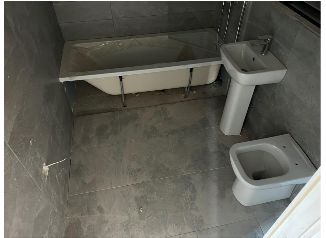
Level 4 – bathroom fittings
