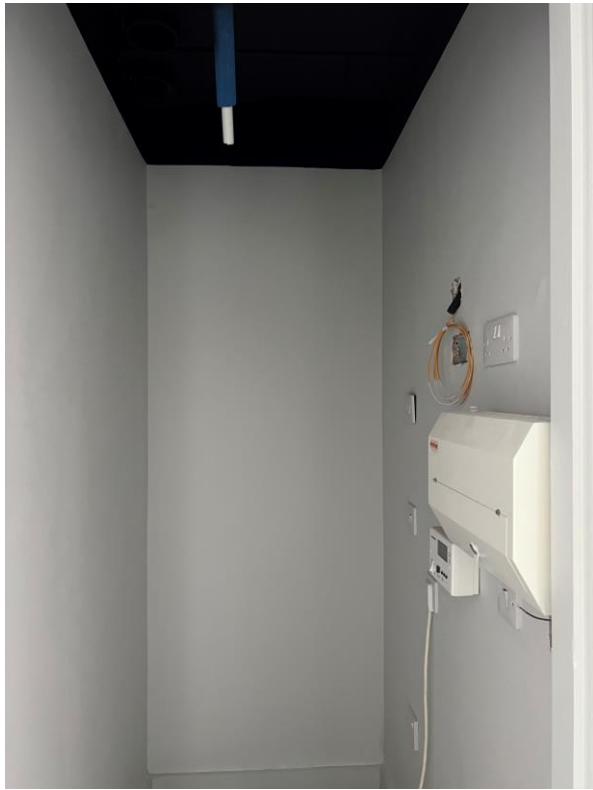
Level 6 – 2 nd fix electrical
