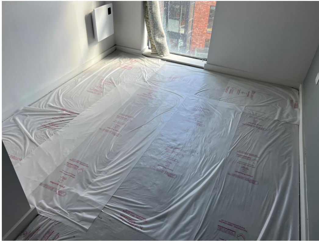
Level 4 – carpet floor covering
