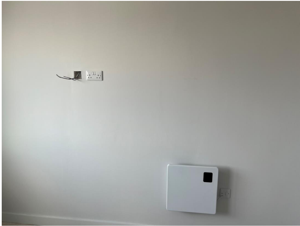
Level 6 – 2 nd fix electrical
