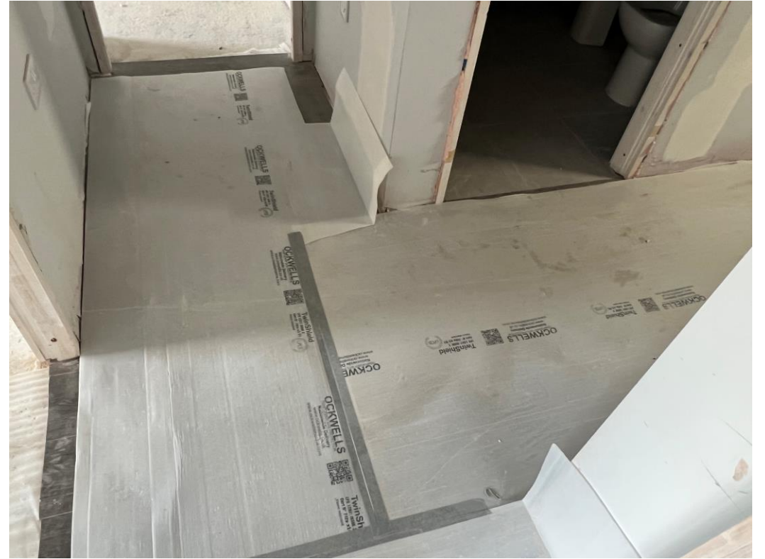
Level 3 – wood laminate flooring
