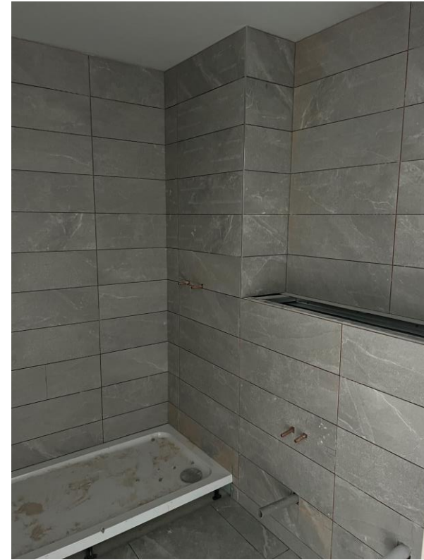
Level 8 – wall and floor tiling
