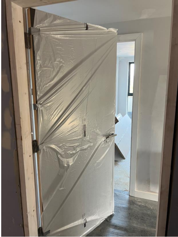
Level 6 – Internal woodgrain doors installed
