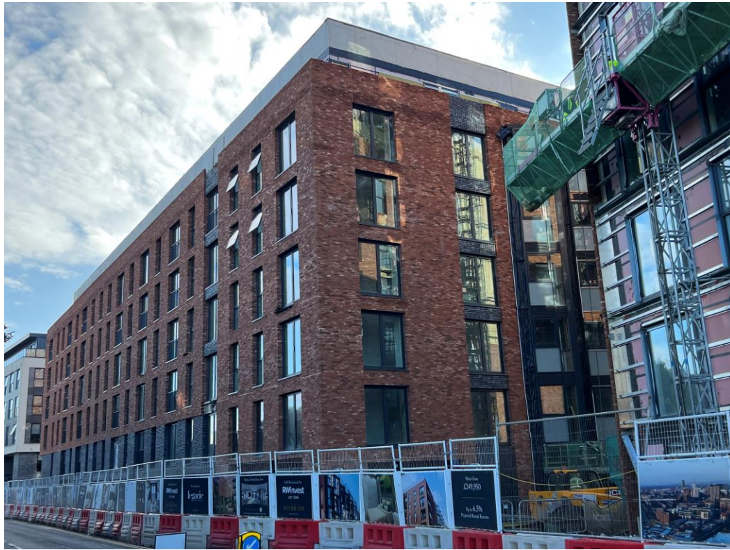
Ordsall Lane site view
