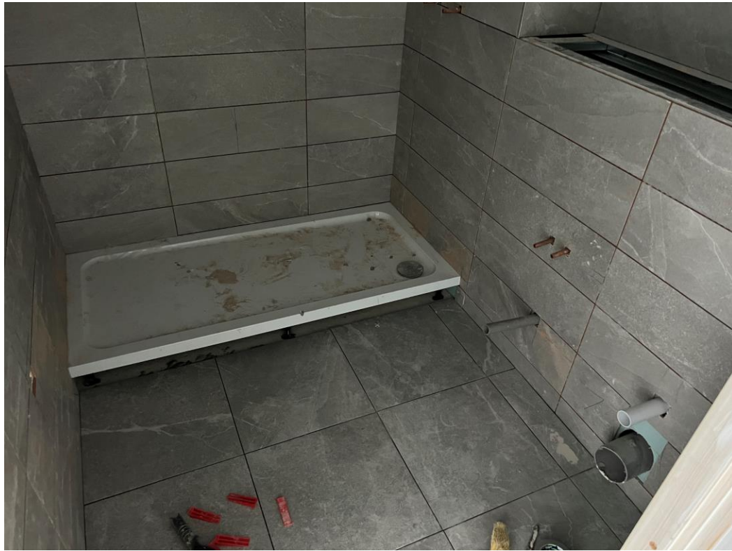
Level 8 – wall and floor tiling
