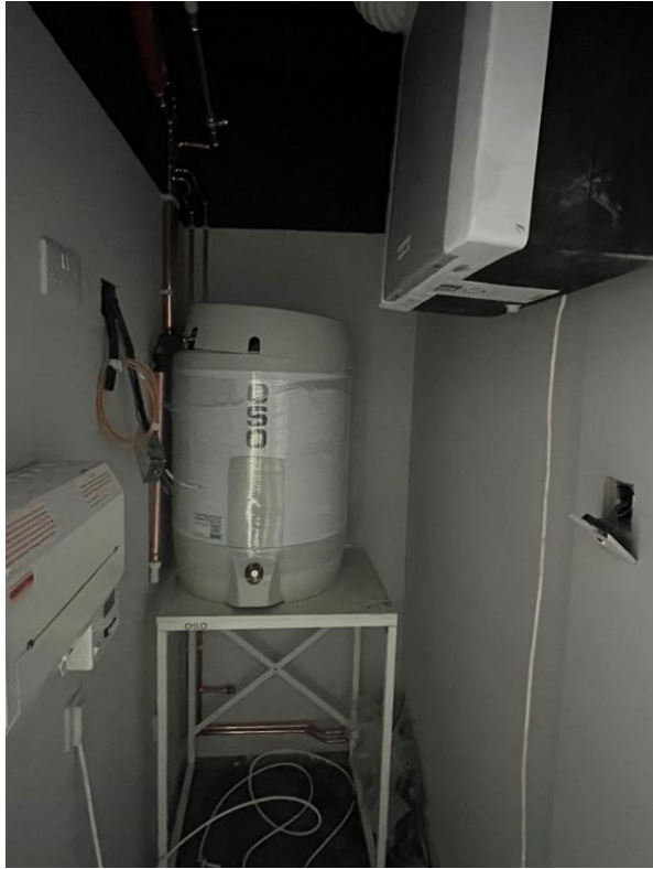
Level 6 – 2 nd fix mechanical
