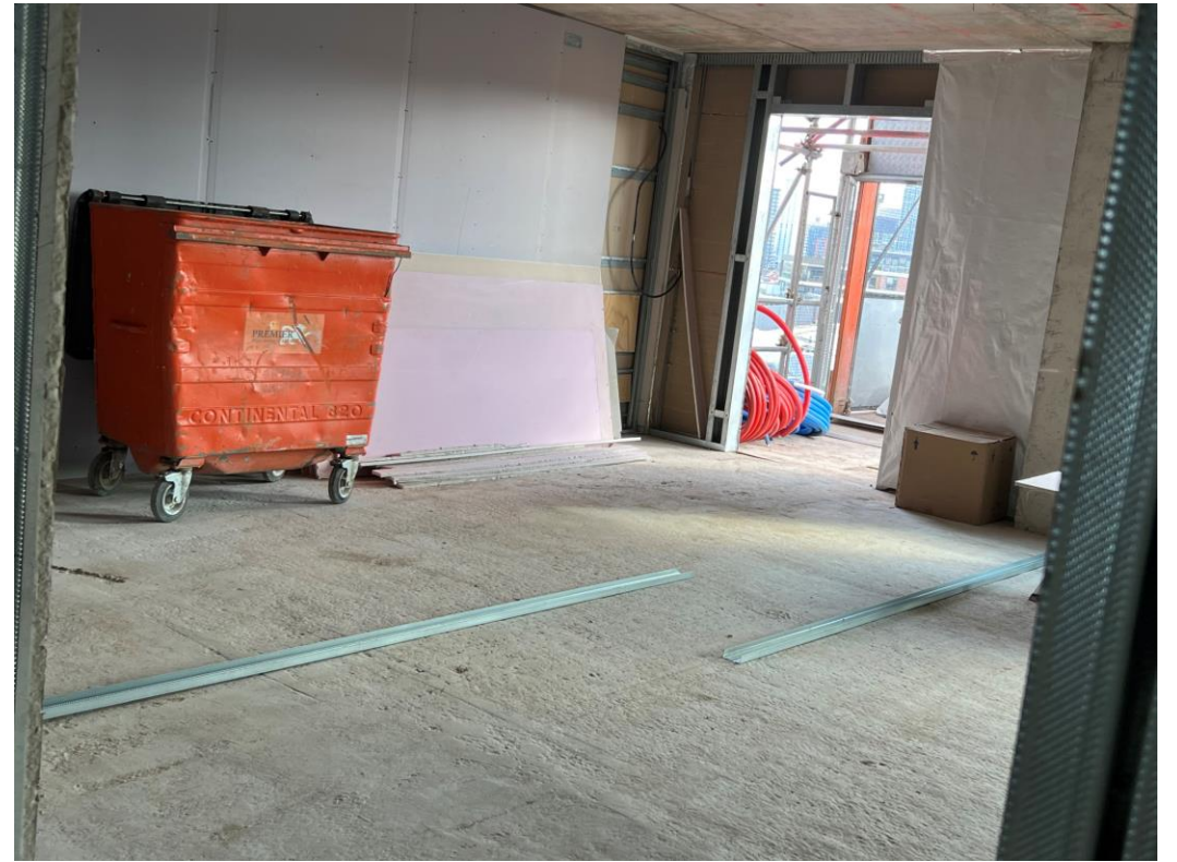
Level 8 – hoist flat setting out partition walls
