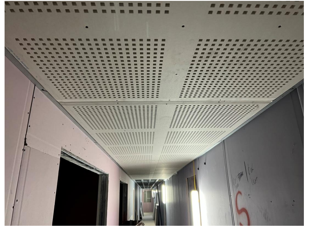
Level 5 – acoustic perforated board to corridor ceiling
