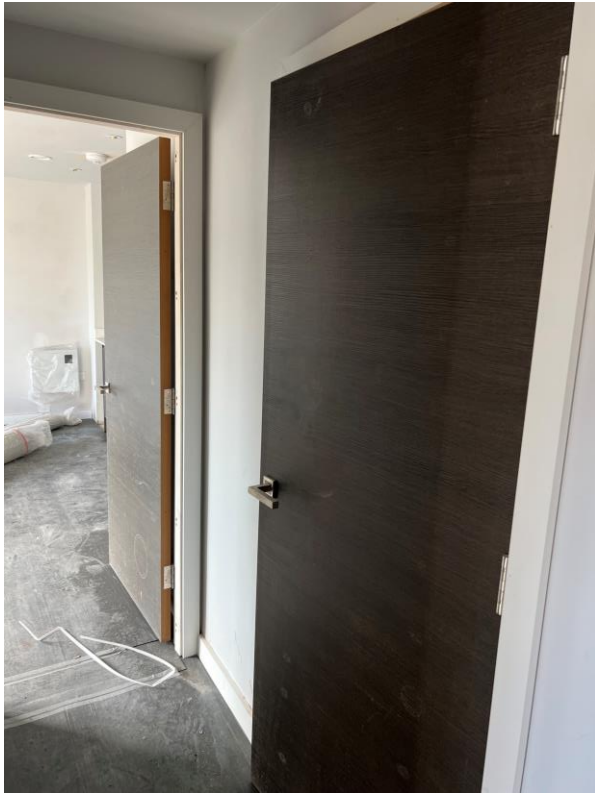
Level 6 – Internal woodgrain doors installed
