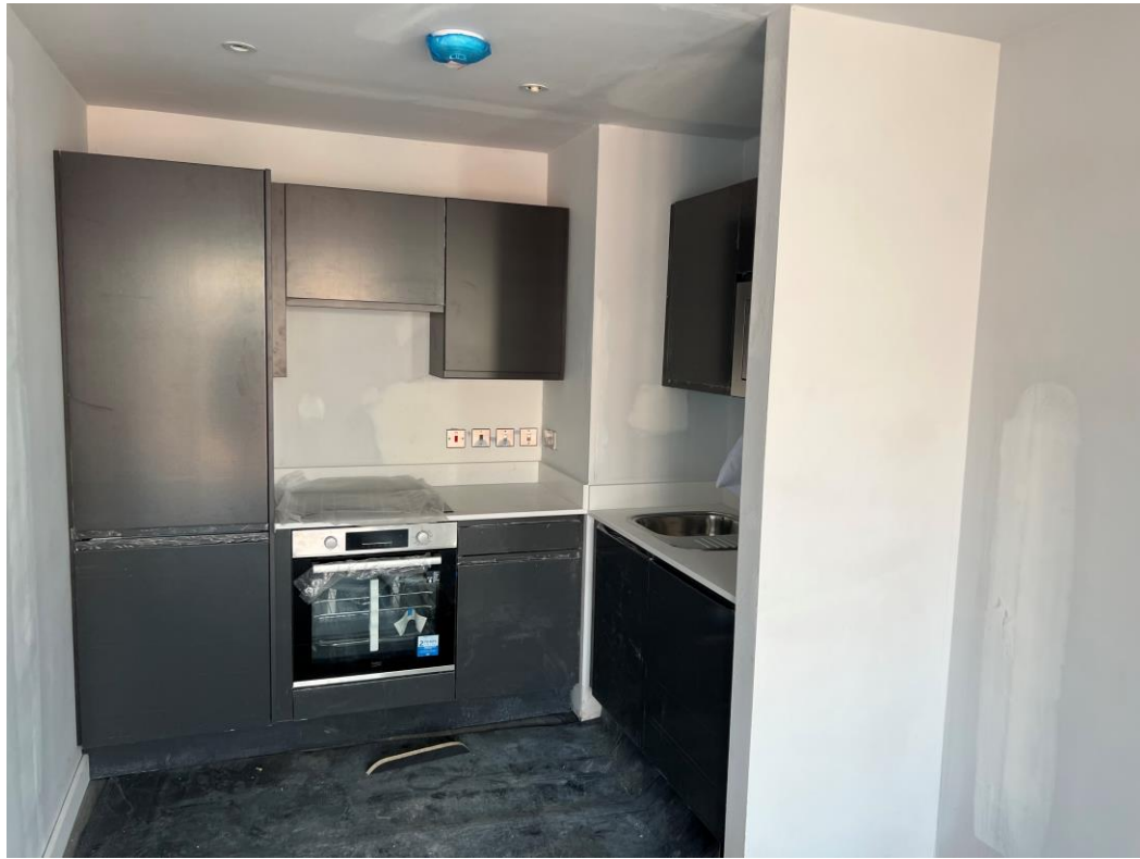
Level 6 – Kitchen units installed
