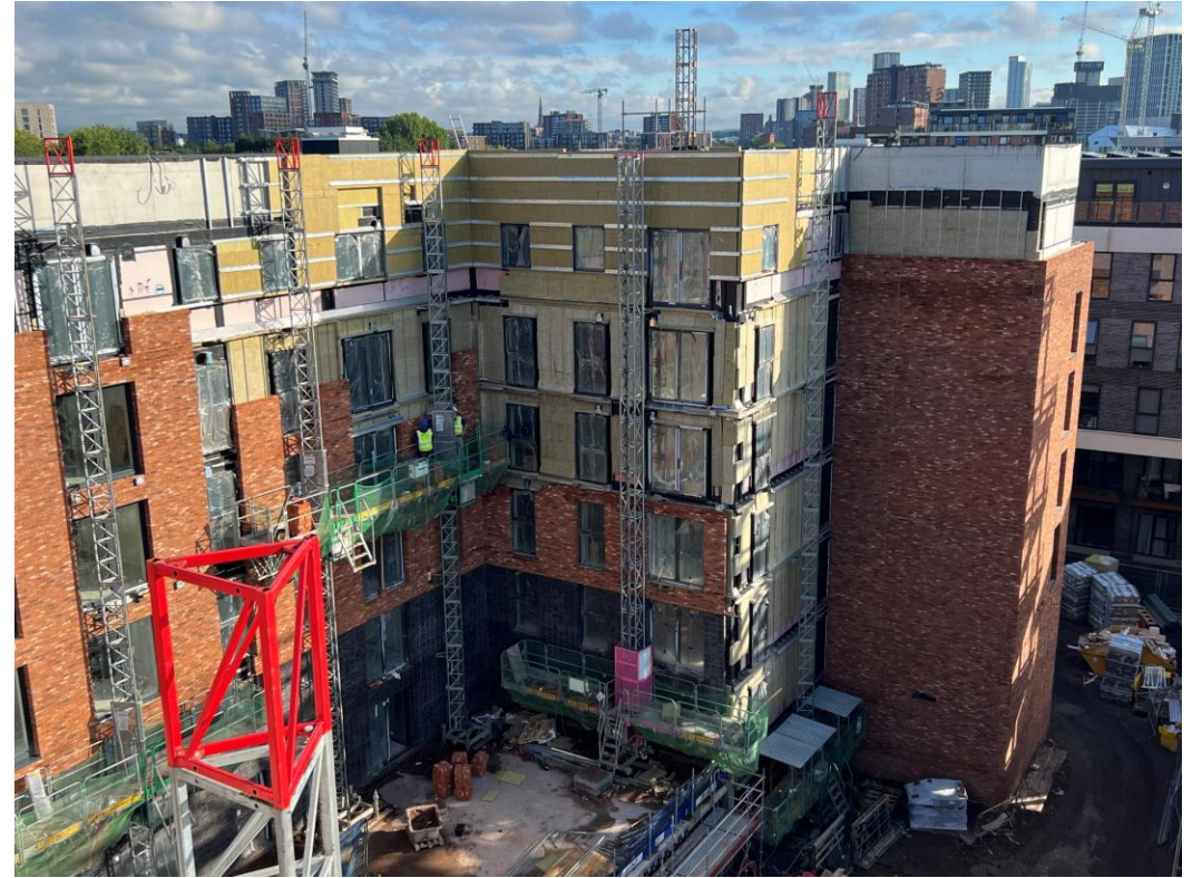
Block B wall insulation and brickwork
