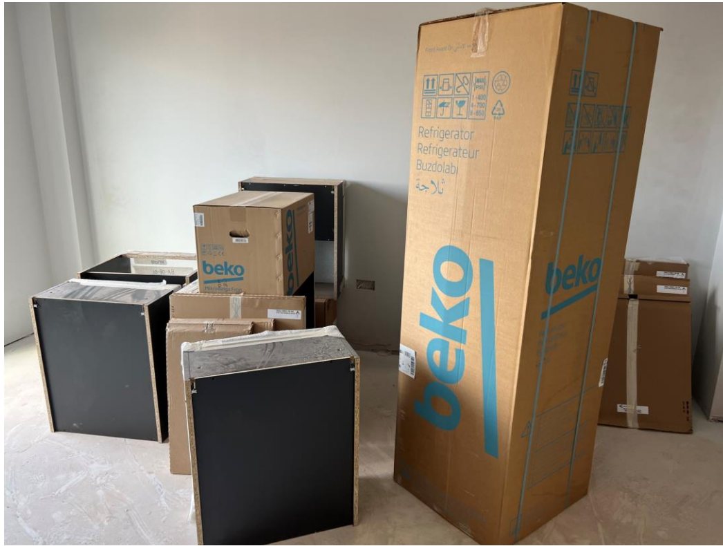
Level 8 – kitchen units loaded for installation
