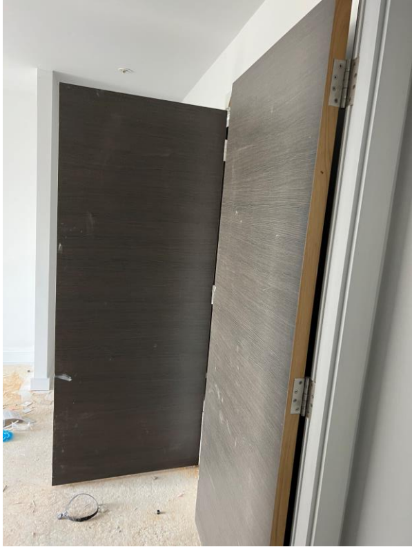
Level 2 – Internal woodgrain doors installed
