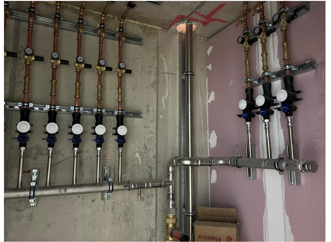
Level 6 – 2 nd fix mechanical installation
