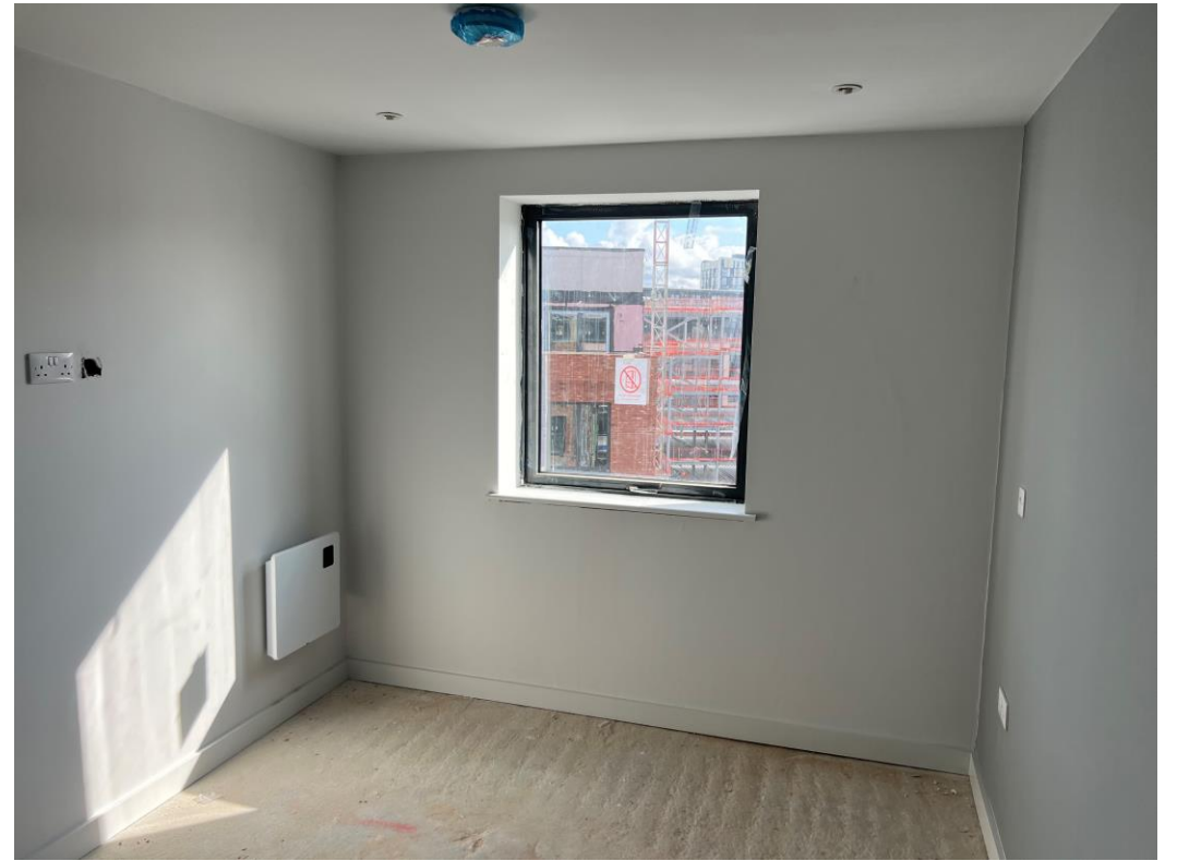
Level 6 – 2 nd fix electrical
