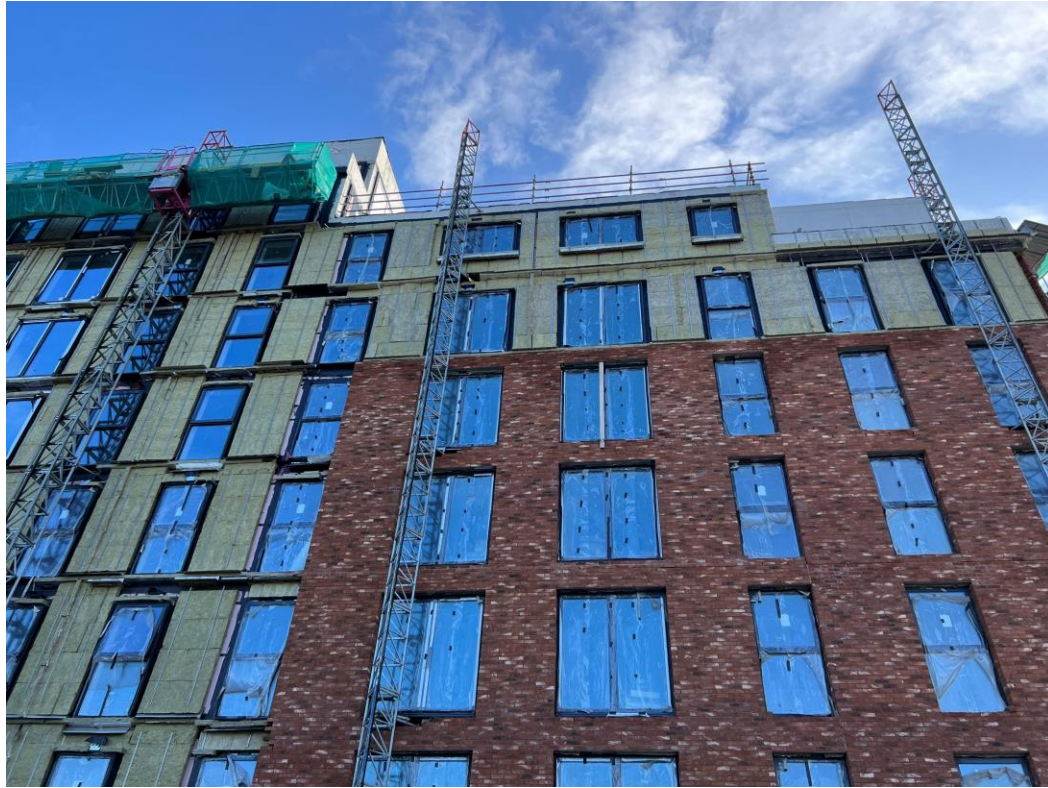
Worrall Street site view
