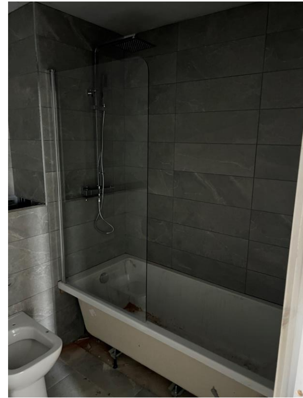
Level 7 – sanitary installation
