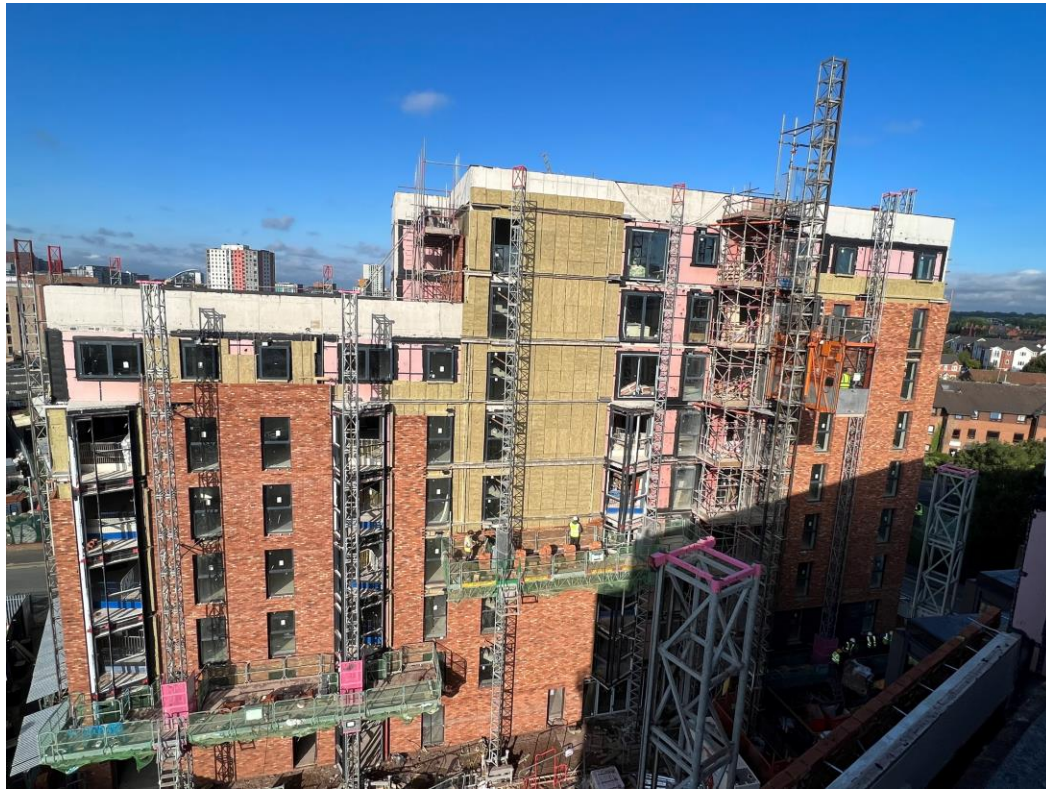
Block A wall insulation and brickwork
