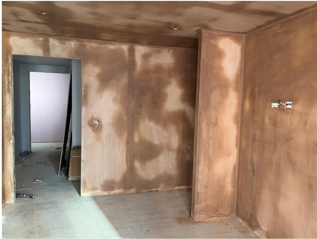
Level 5 – walls and ceiling plaster skim finish
