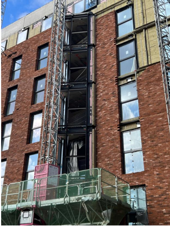
Block A curtain walling
