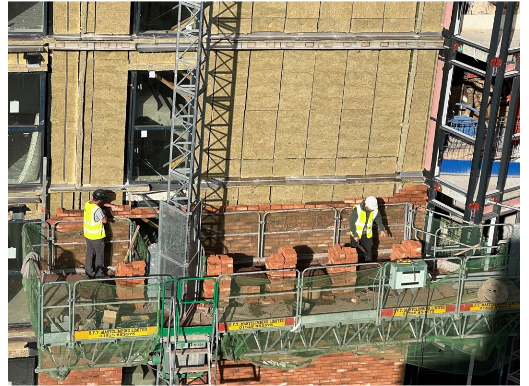
Block A wall insulation and brickwork
