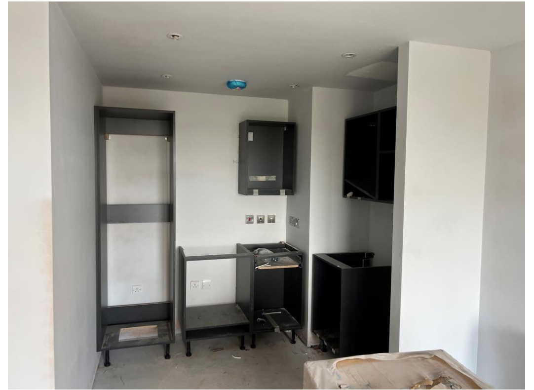
Level 7 – Kitchen units installed
