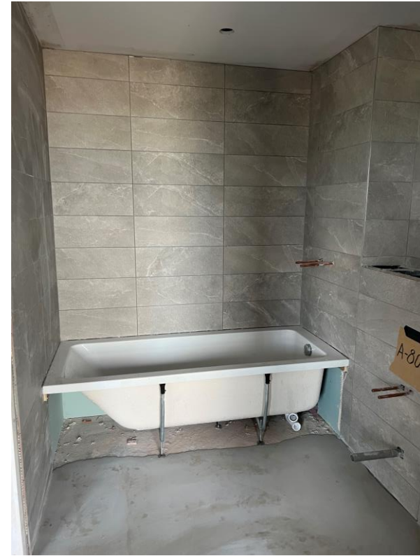
Level 8 – wall and floor tiling
