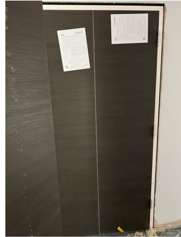
Level 6 – Internal woodgrain doors installed
