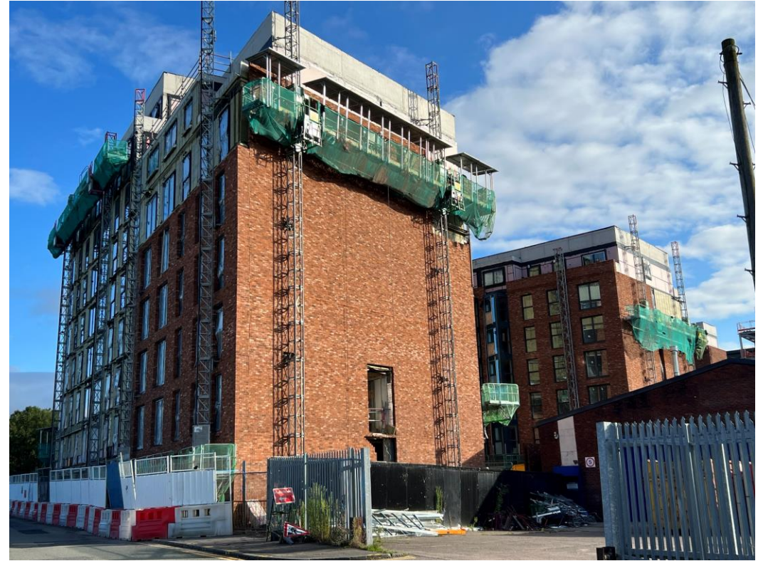
Worrall Street site view
