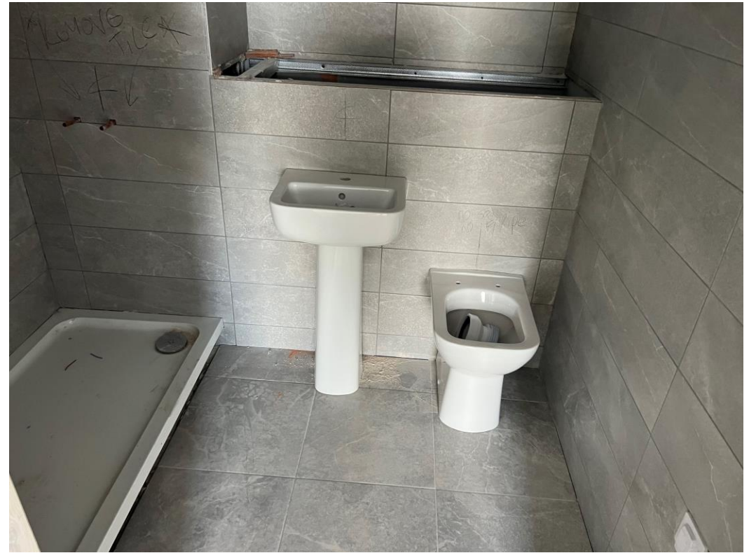
Level 7 – sanitary installation
