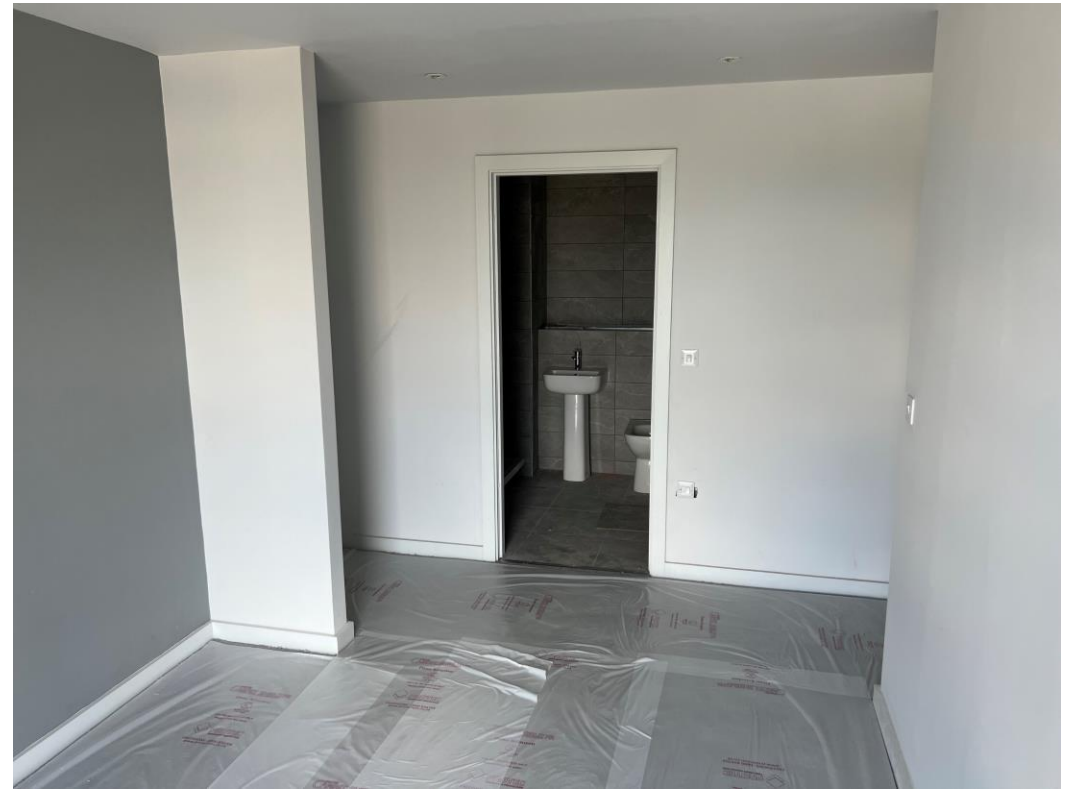
Level 4 – carpet floor covering
