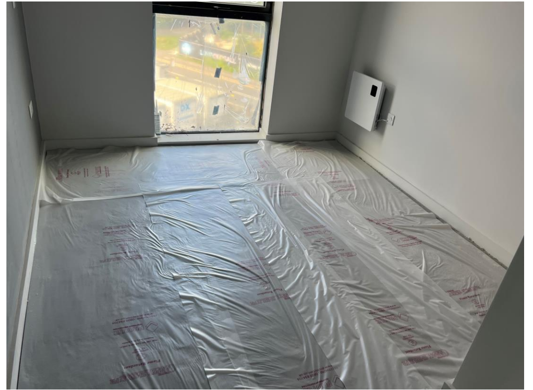
Level 4 – carpet floor covering
