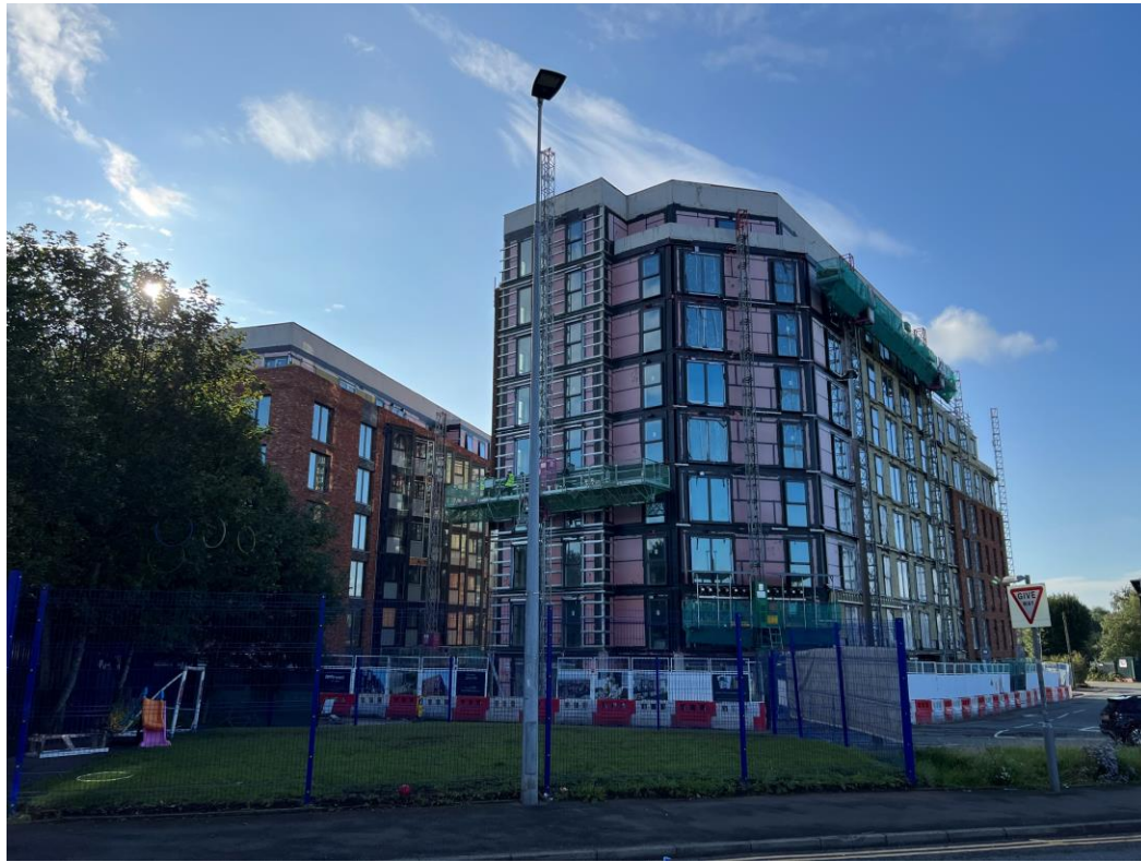
Ordsall Lane site view
