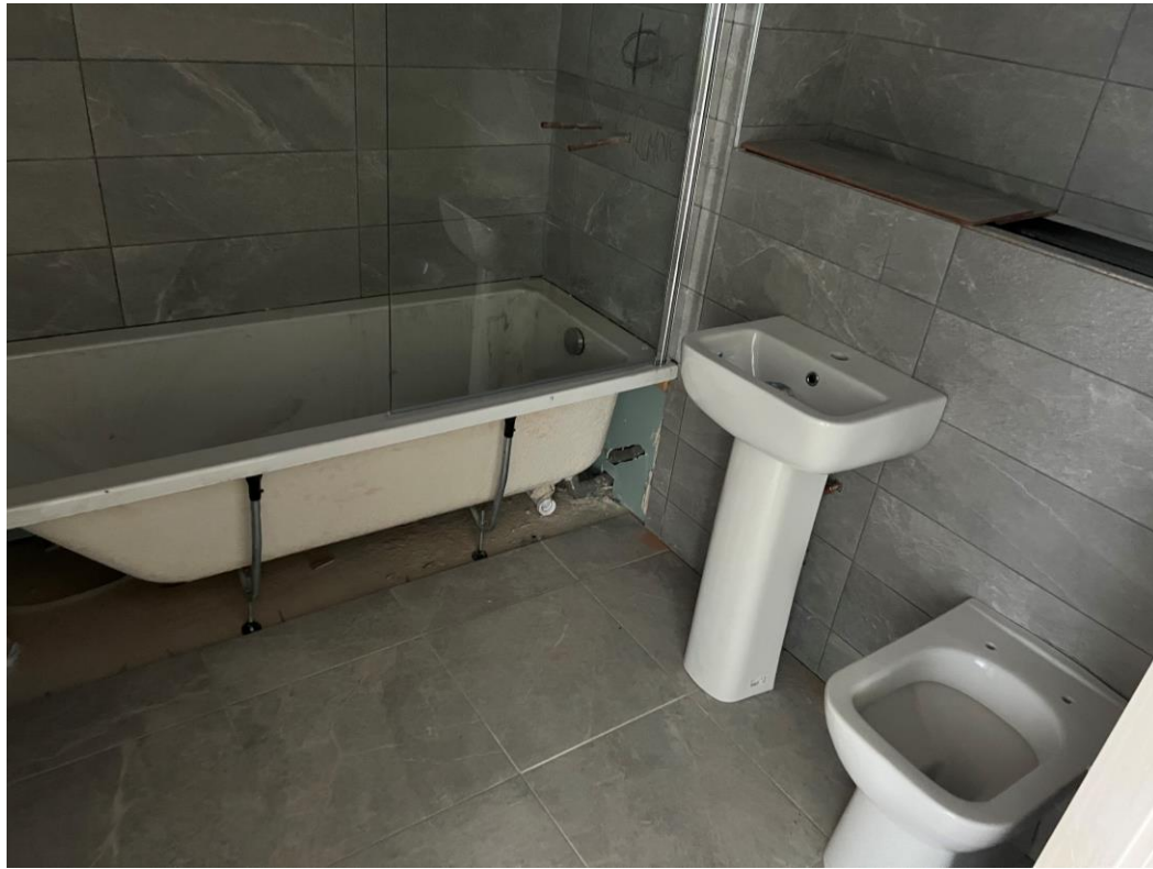
Level 7 – sanitary installation
