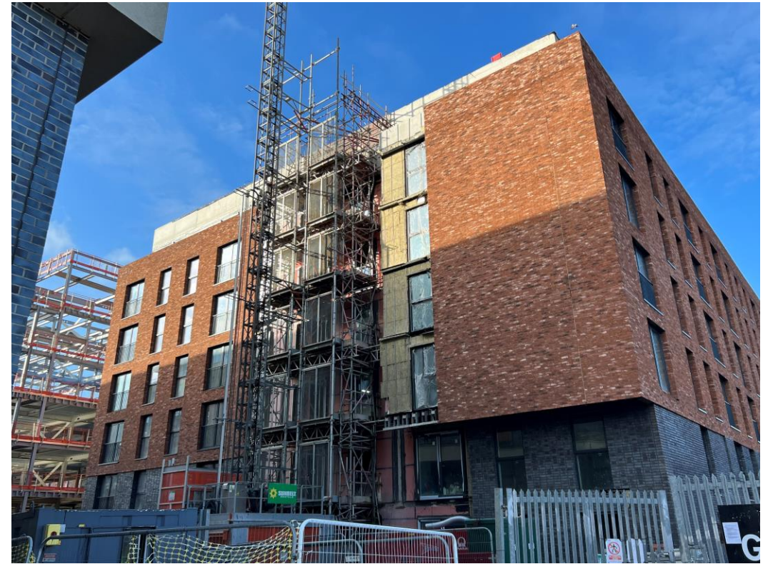
Ordsall Lane site view
