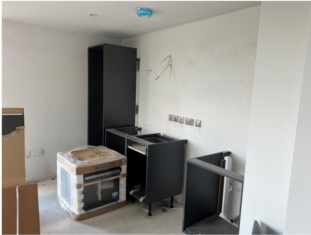
Level 7 – Kitchen units installed
