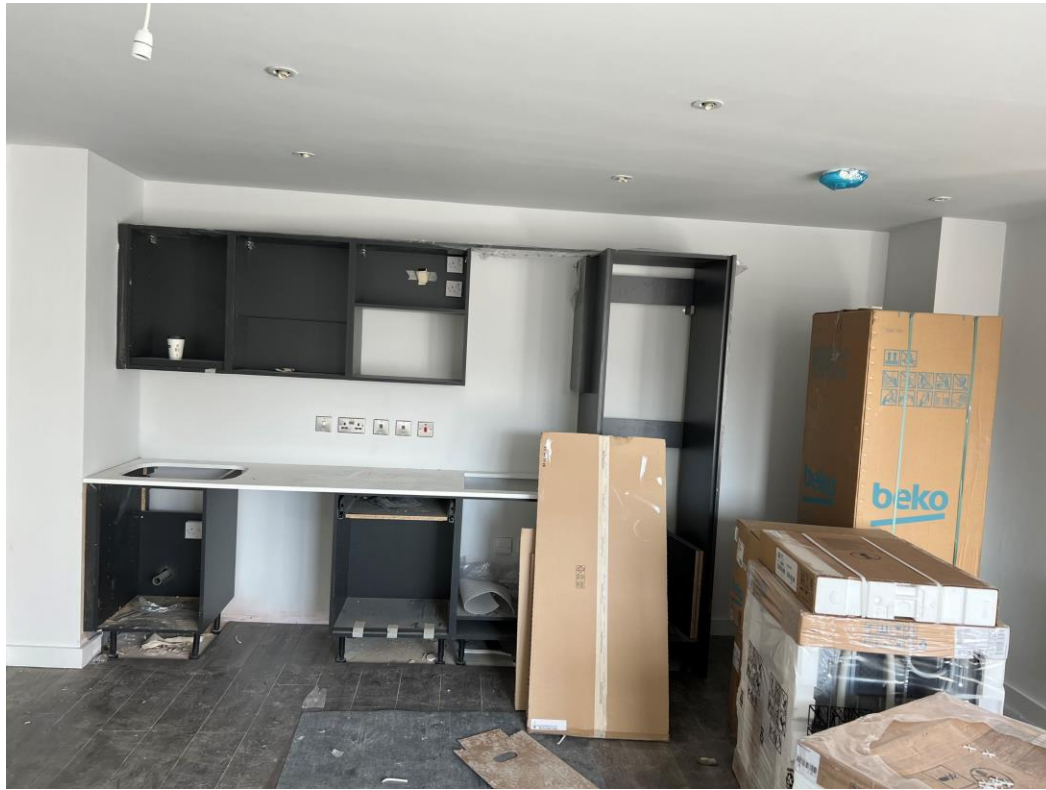
Level 6 – Kitchen units installed
