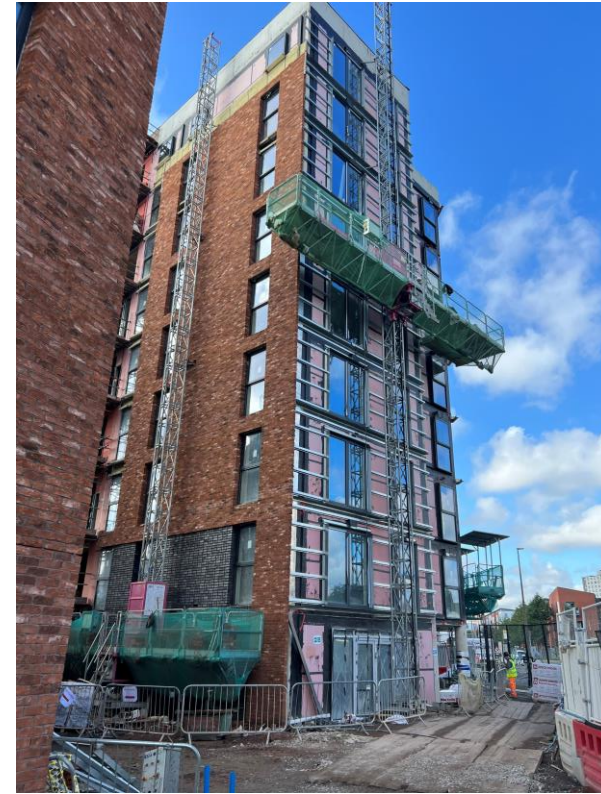
Block A wall insulation and brickwork
