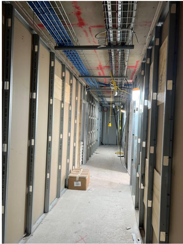
Level 8 – corridor walls formed
