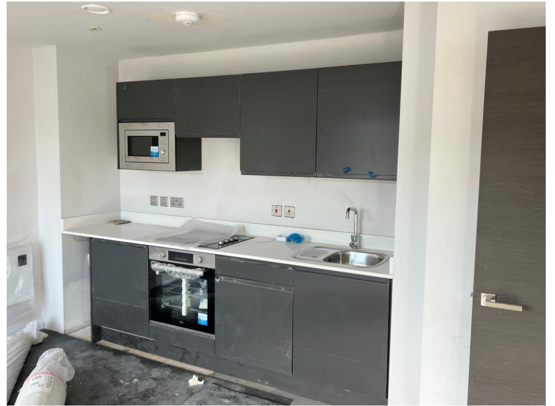
Level 6 – Kitchen units installed
