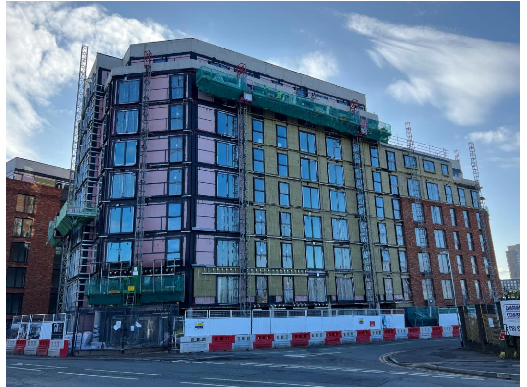
Ordsall Lane site view
