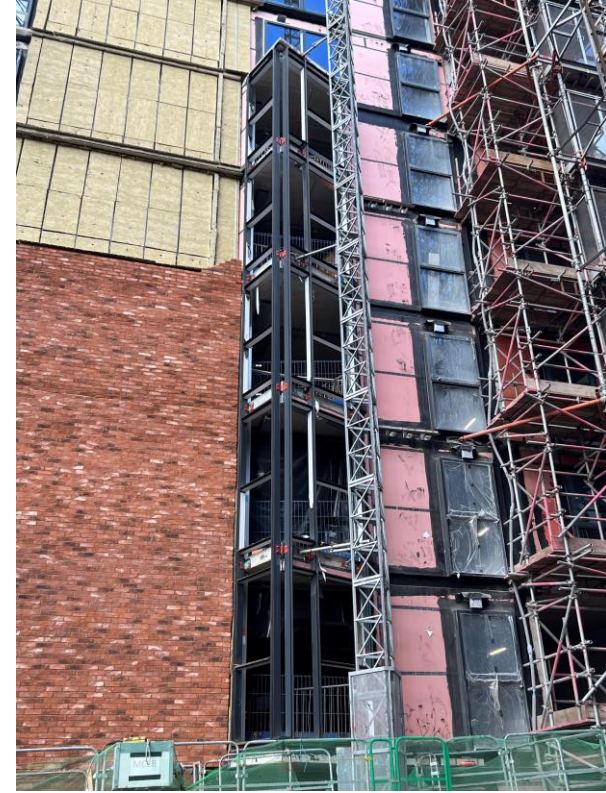
Block A curtain walling
