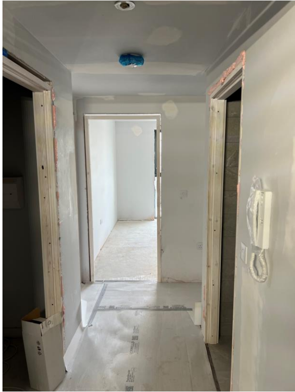
Level 3 – wood laminate flooring
