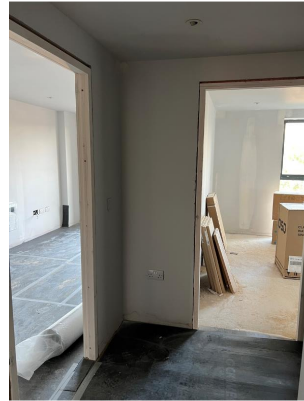
Level 5 – wood laminate flooring
