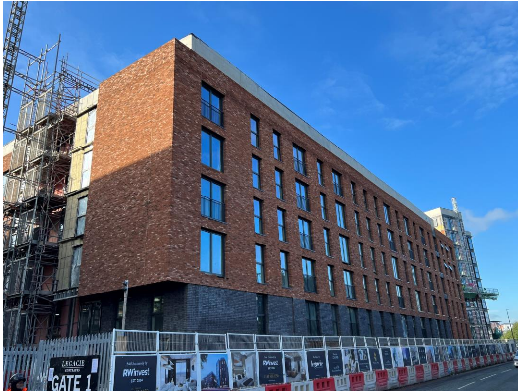
Ordsall Lane site view
