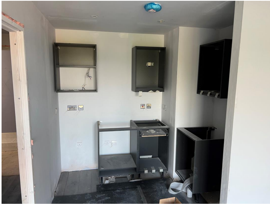
Level 5 – Kitchen units installed
