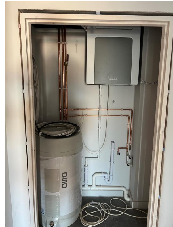
Level 3 – 2 nd fix mechanical
