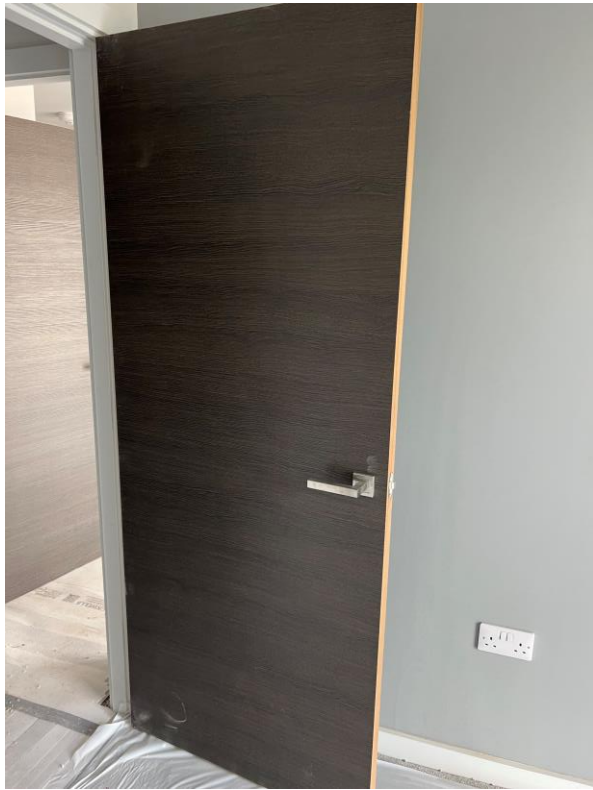
Level 1 – Internal woodgrain doors installed
