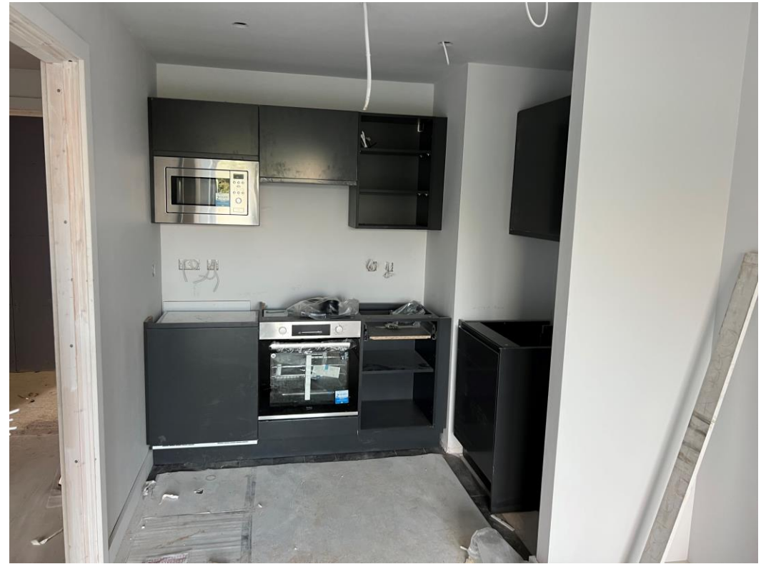
Level 5 – Kitchen units installed
