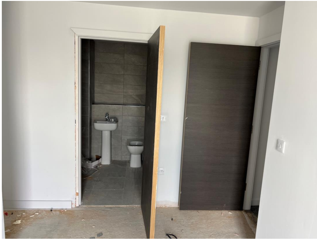
Level 2 – Internal woodgrain doors installed
