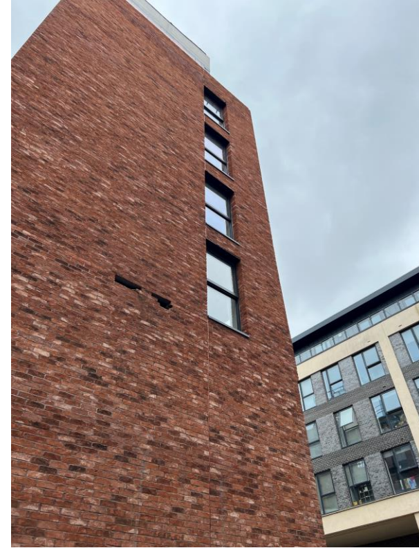
Block B wall insulation and brickwork
