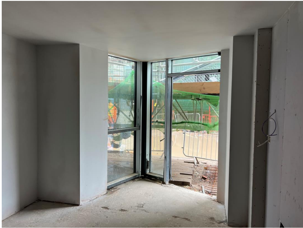
Ground Level 1 – Apartments formed
