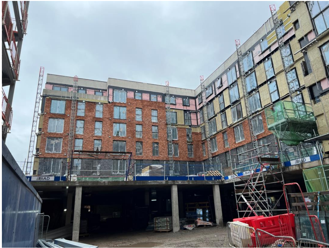
Block B wall insulation and brickwork
