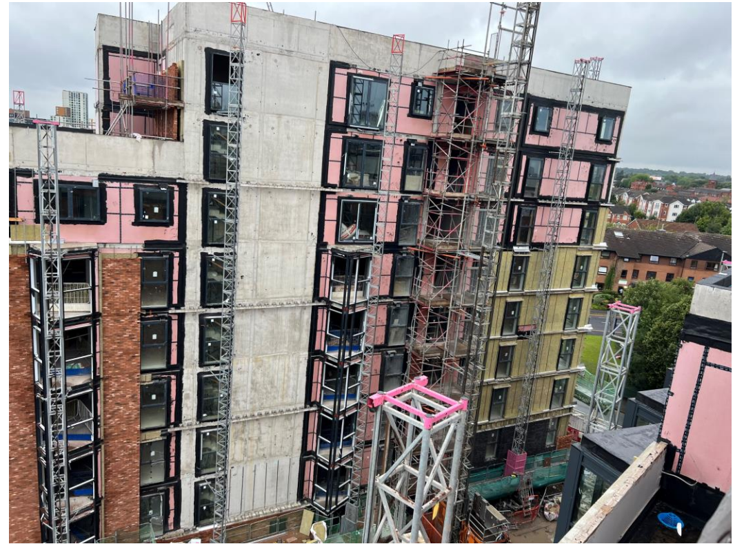
Block A wall insulation and brickwork
