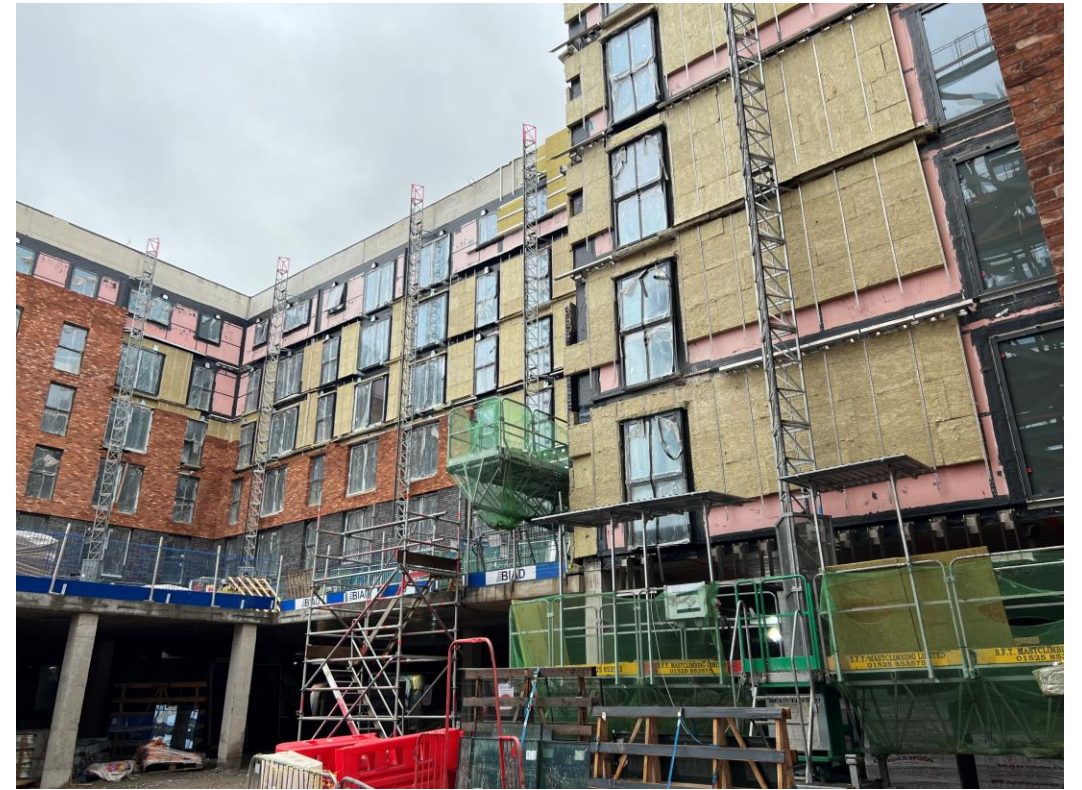
Block B wall insulation and brickwork
