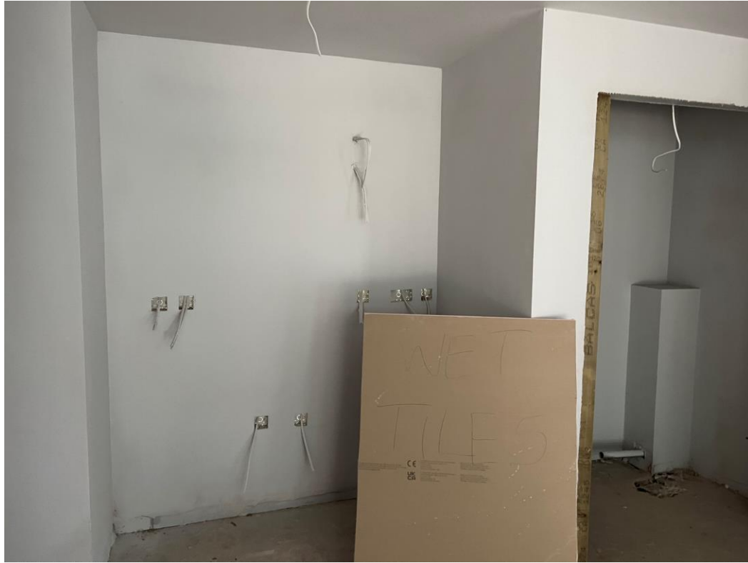
Ground Level 1 – Apartments formed
