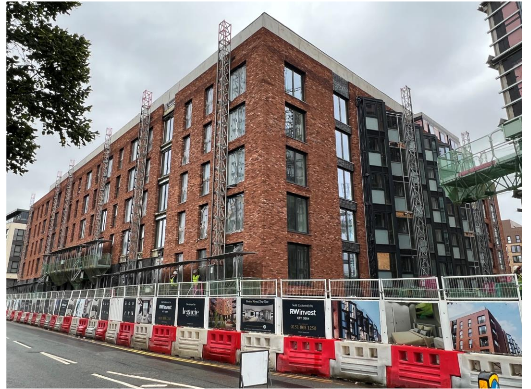
Ordsall Lane site view
