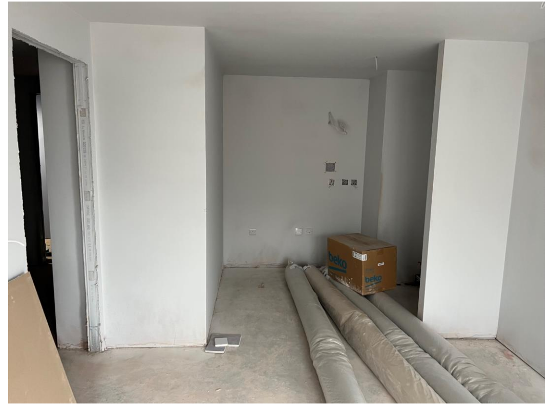
Level 5 – Carpet floor covering loaded for installation
