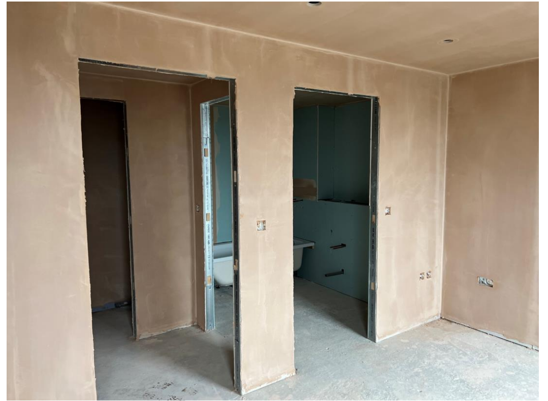
Level 8 – walls and ceilings plastered
