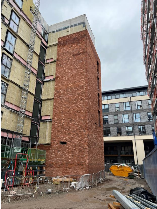
Block B wall insulation and brickwork
