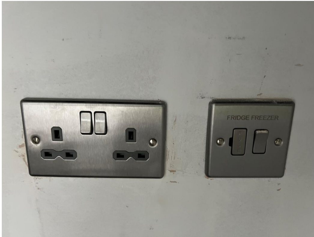
Level 2 – 2 nd fix electrical sockets
