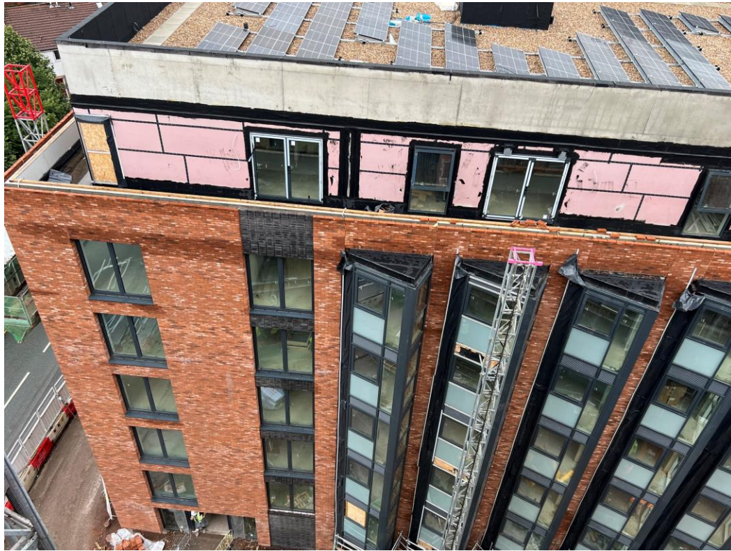
Block B Curtain walling and brickwork
