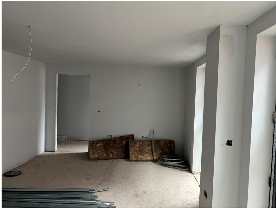
Ground Level 1 – Apartments formed
