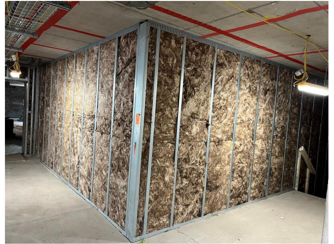
Ground Level 1 – Apartments formed
