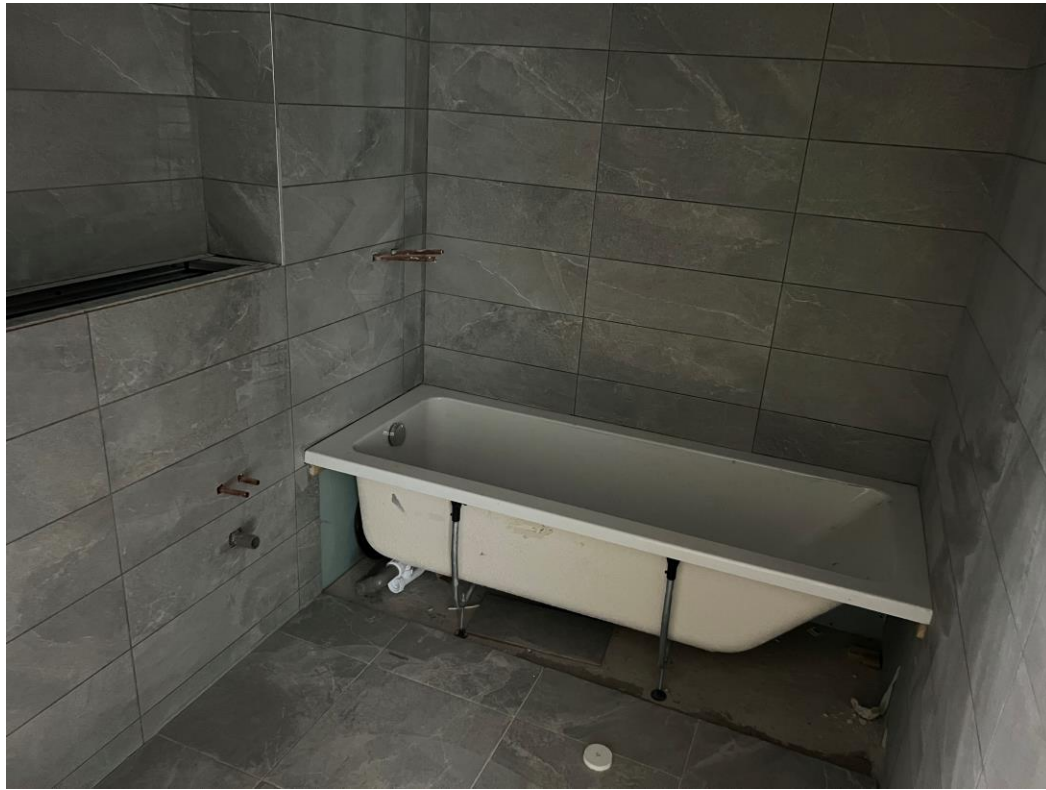
Level 7 – wall and floor tiling
