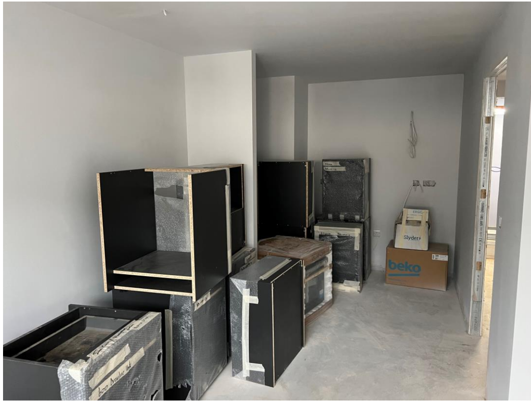
Level 5 – Kitchen units loaded for installation
