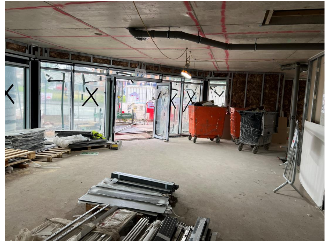
Ground Level – commercial unit
