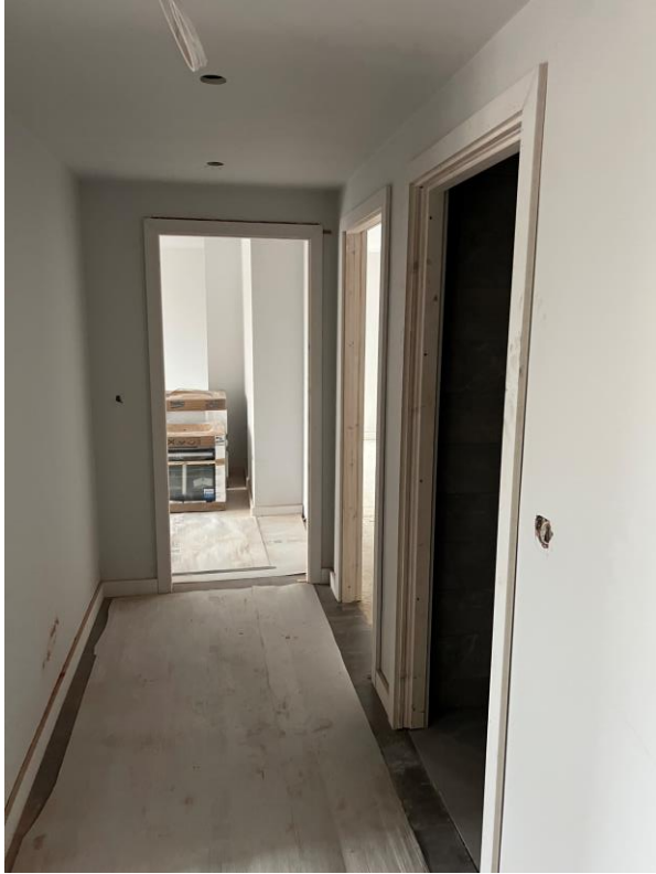
Level 4 – doorcasings, skirting and architrave
