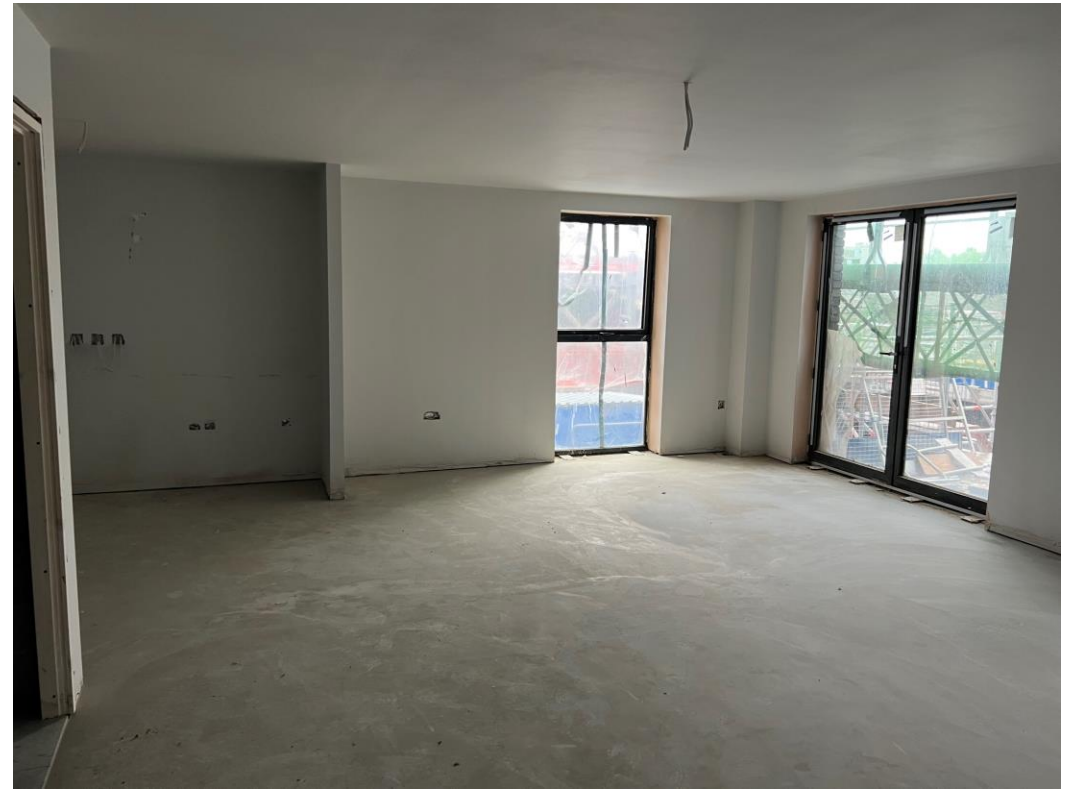
Level 1 – latex screed floors
