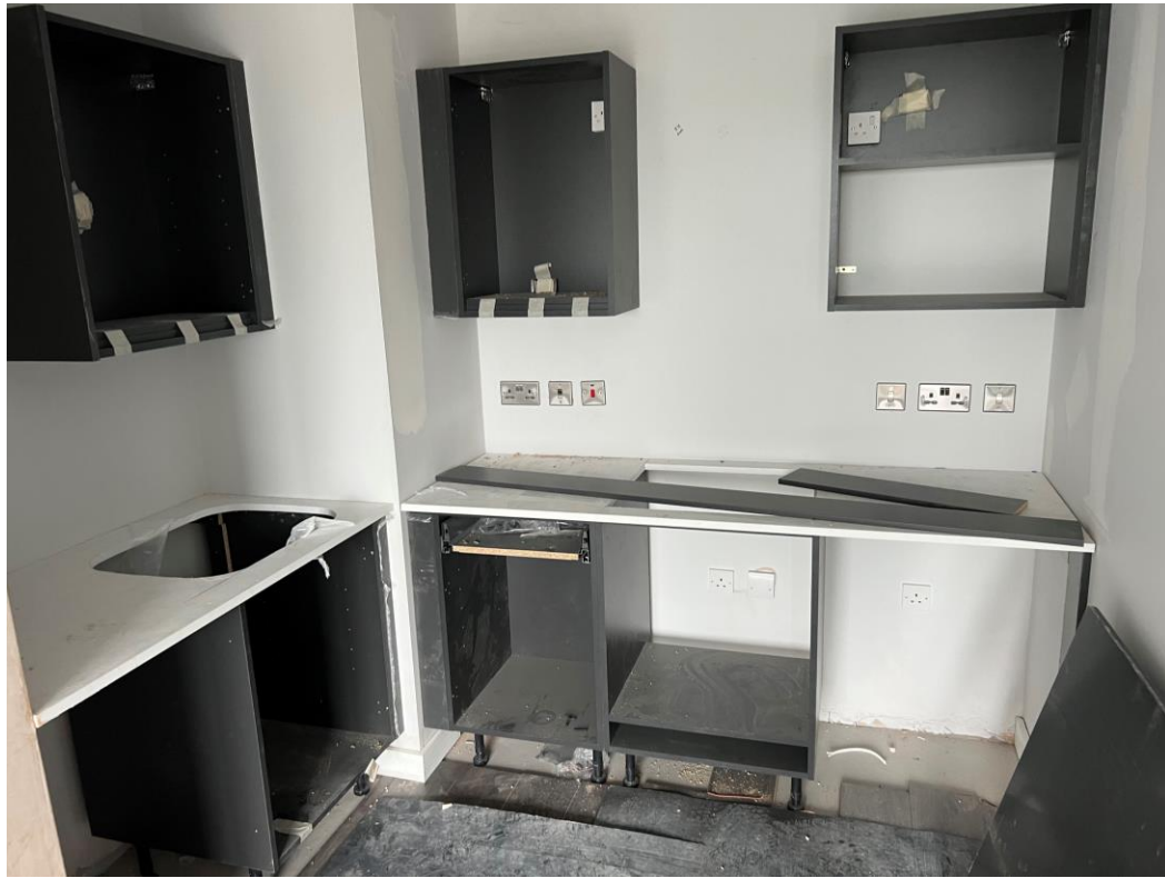
Level 6 – Kitchen units installed
