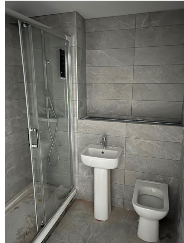
Level 3 – Bathroom fittings installed
