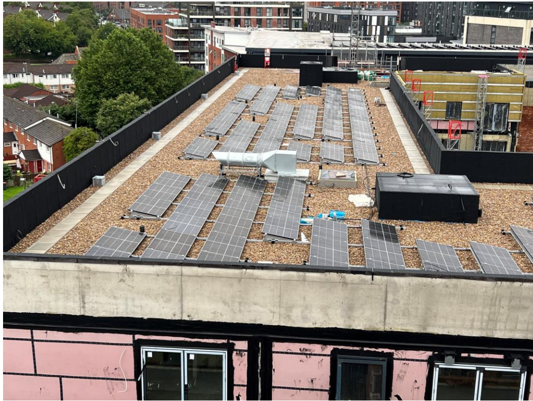
Block B inverted main roof system complete
