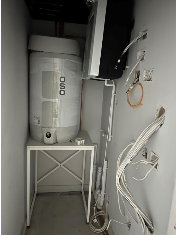
Level 3 – 2 nd fix mechanical
