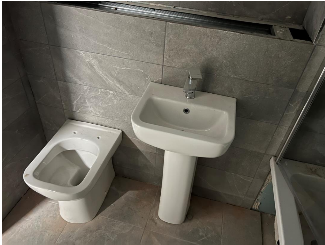
Level 3 – Bathroom fittings installed
