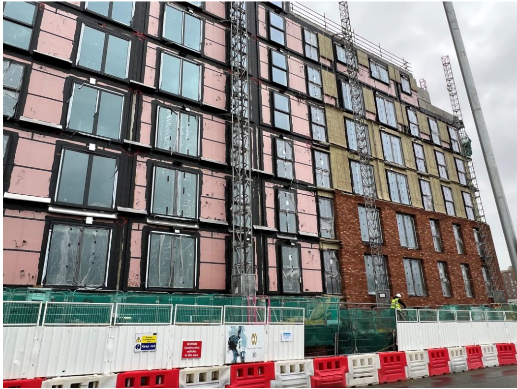
Worrall Street site view
