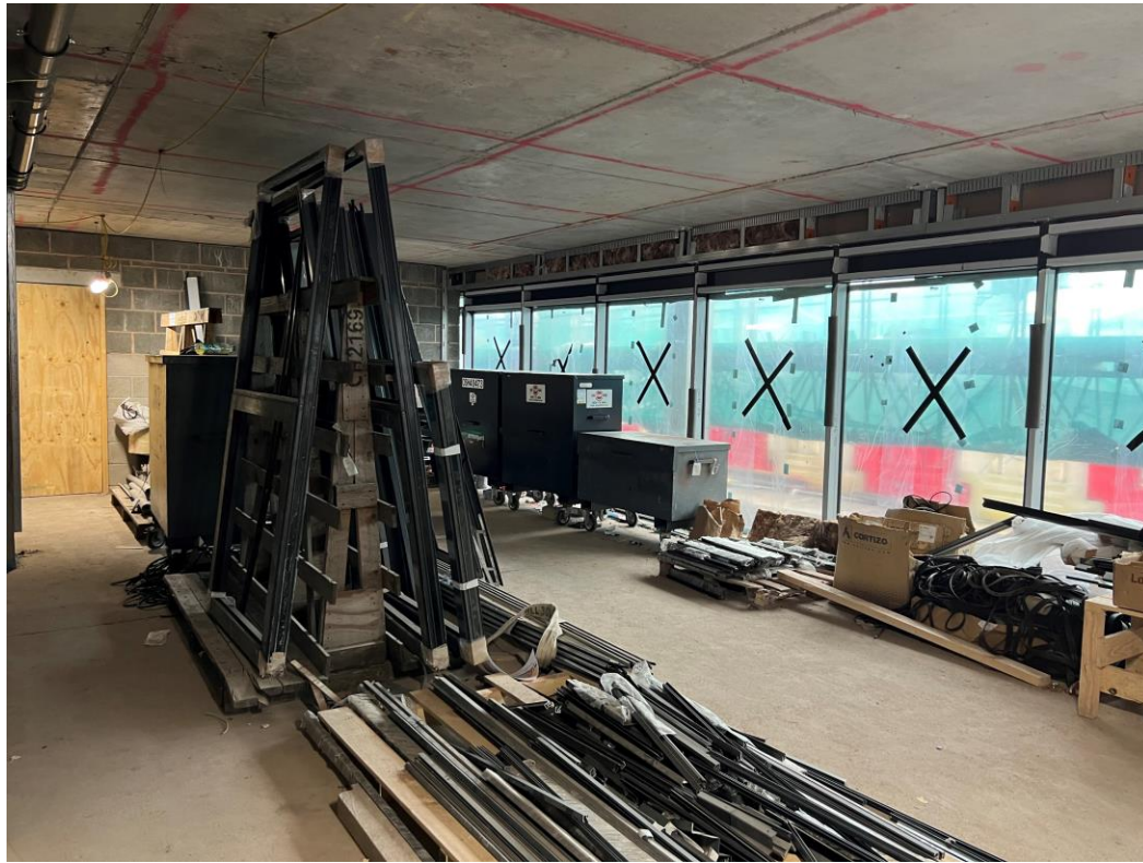
Ground Level – commercial unit
