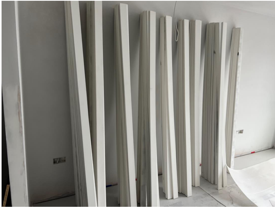
Level 6 – doorcasings, skirting and architrave
