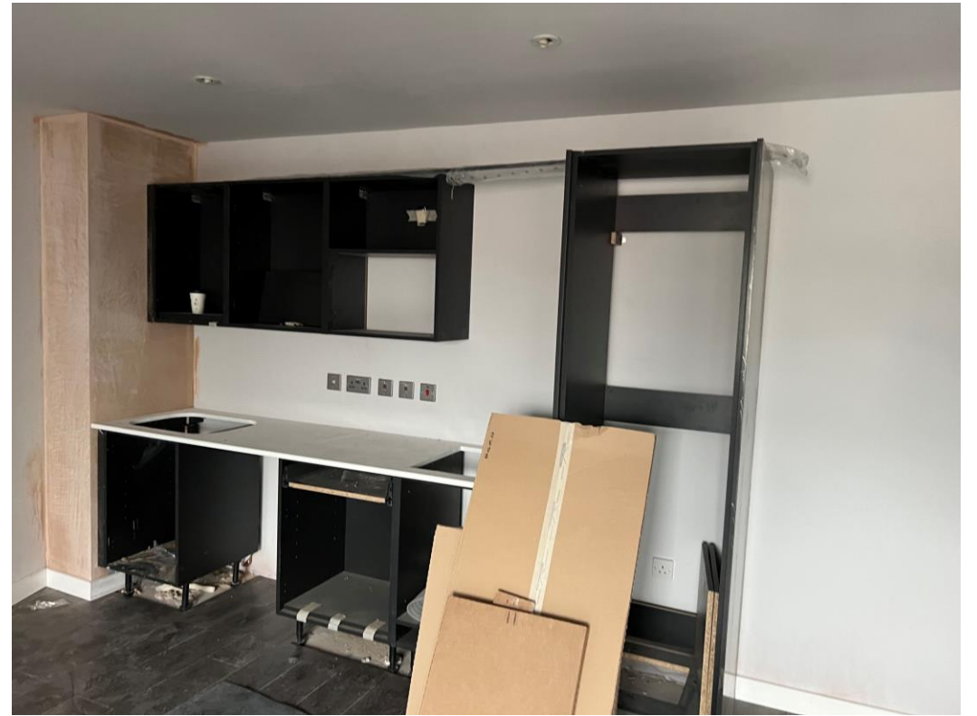
Level 6 – Kitchen units installed
