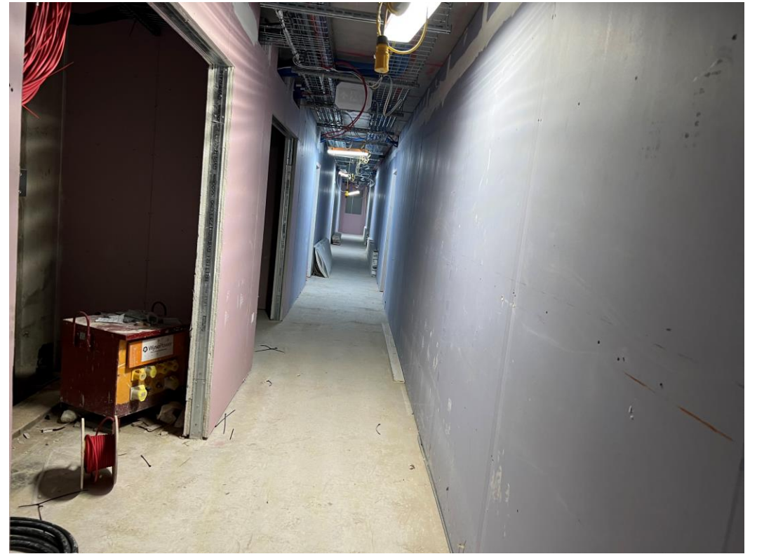
Level 6 – corridor and apartment walls formed
