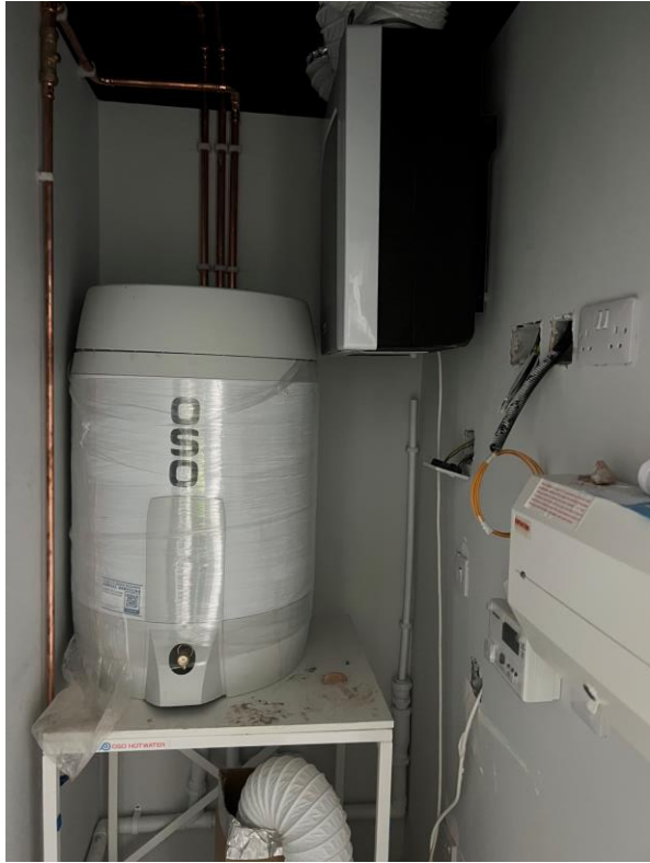
Level 5 – 2 nd fix mechanical installation
