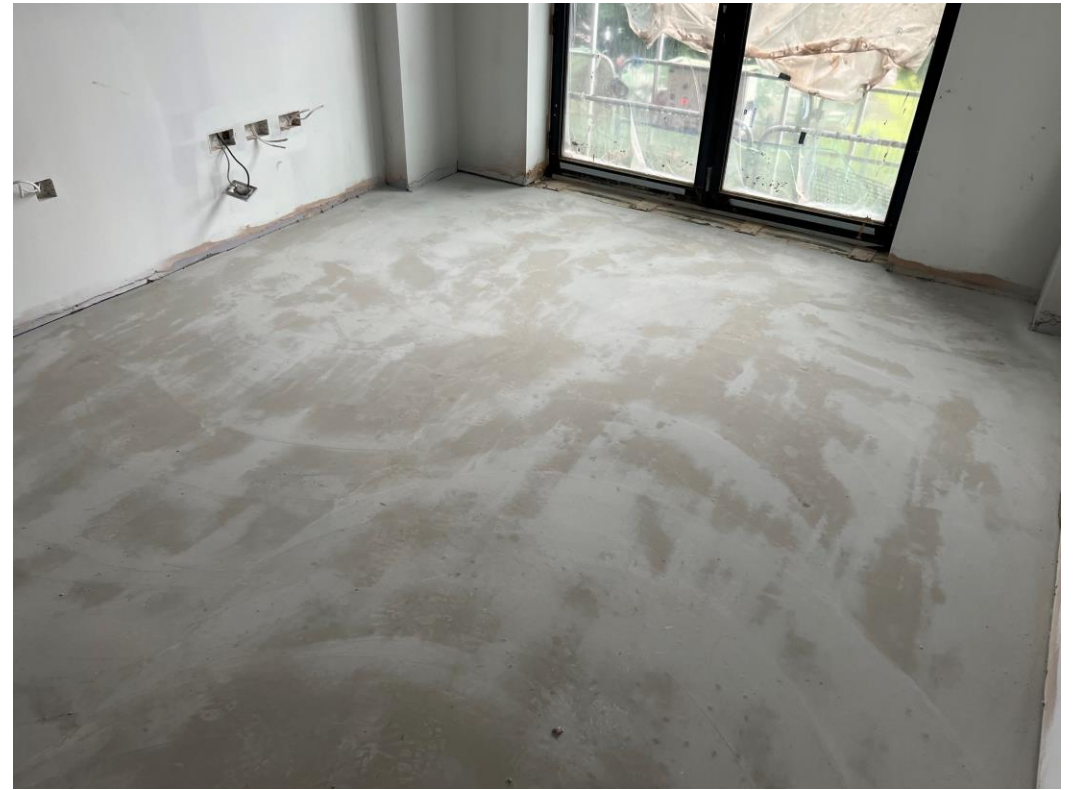
Level 2 – latex screed floors
