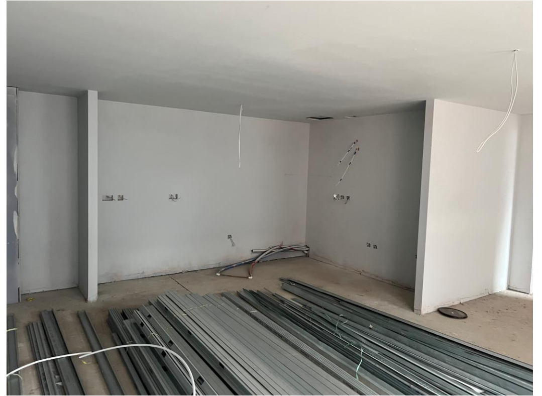
Ground Level 1 – Apartments formed
