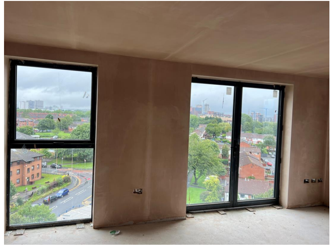
Level 8 – walls and ceilings plastered
