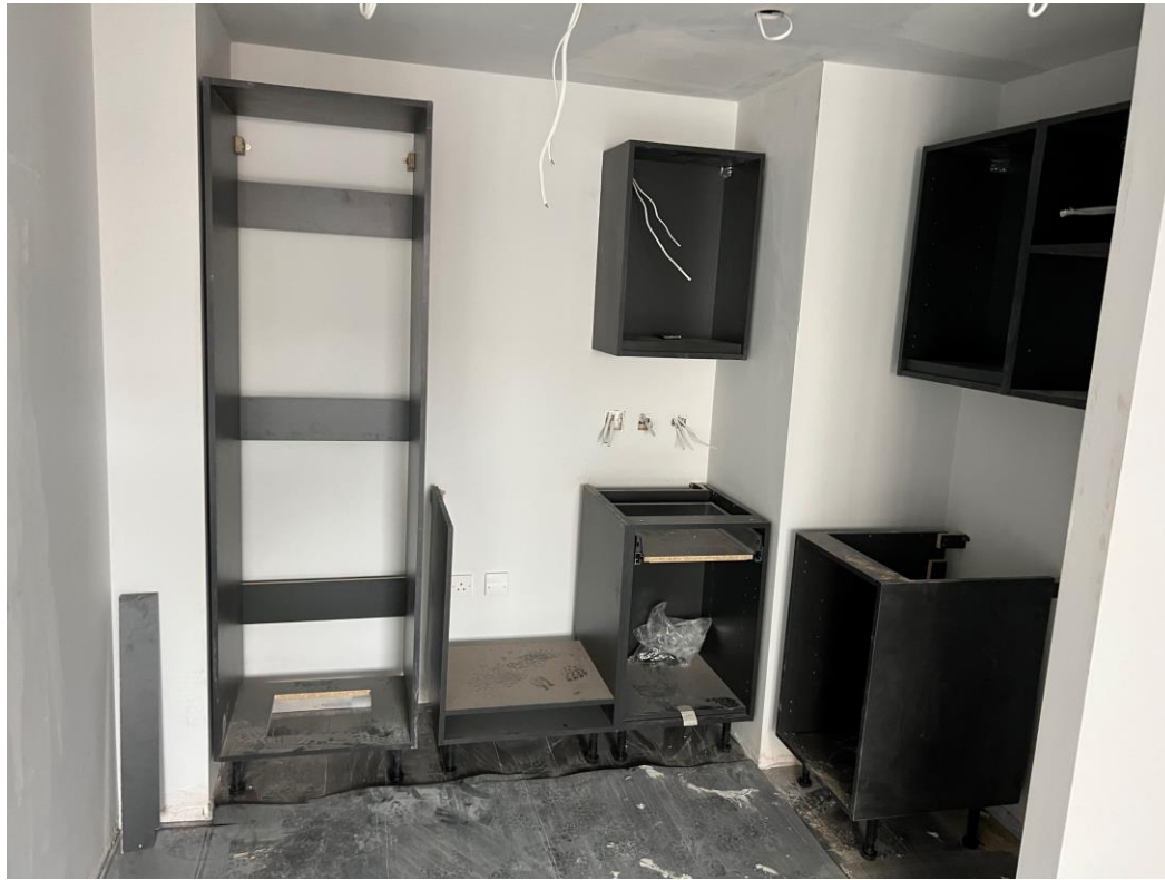
Level 6 – Kitchen units installed
