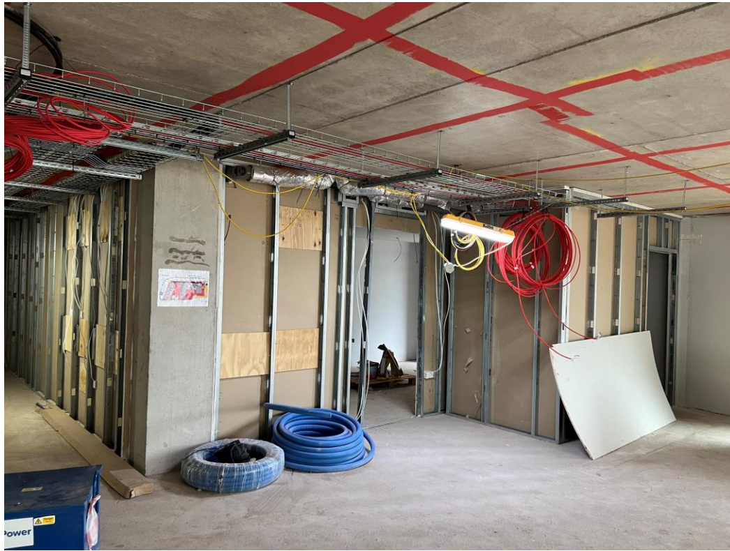
Ground Level 1 – Apartments formed
