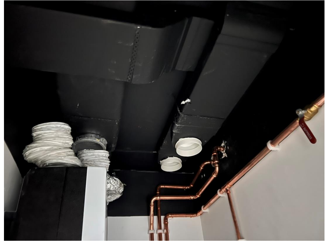
Level 2 – 2 nd fix mechanical
