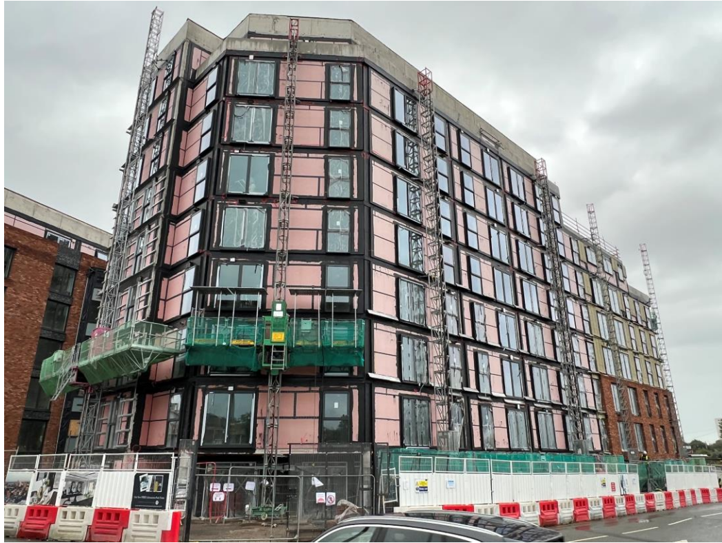
Ordsall Lane site view
