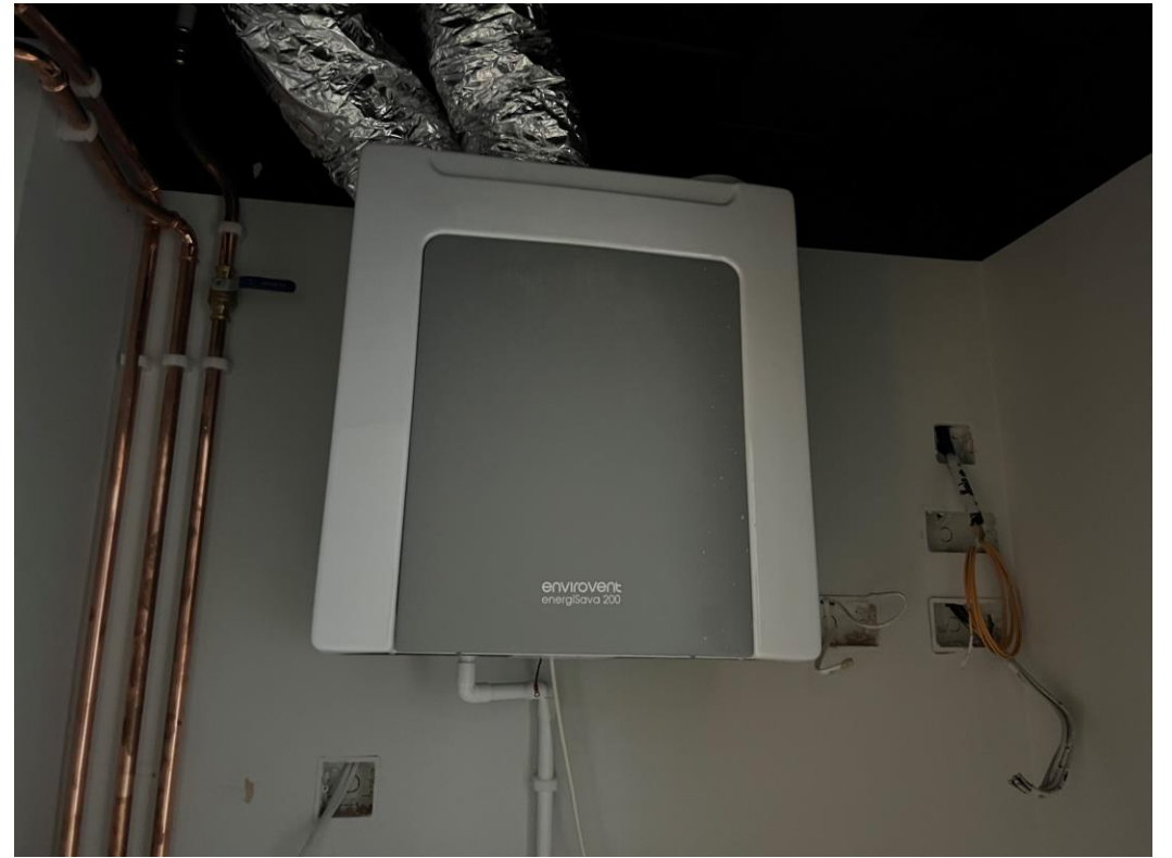
Level 3 – 2 nd fix mechanical
