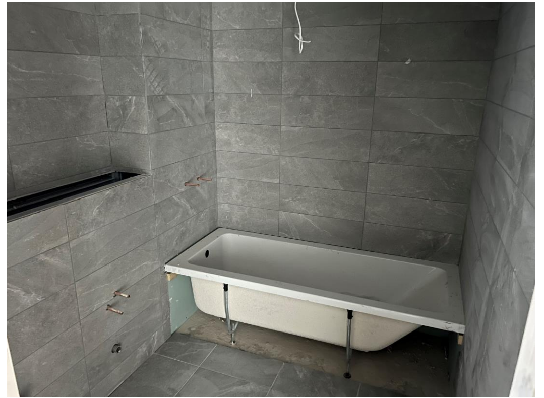
Level 6 – wall and floor tiling
