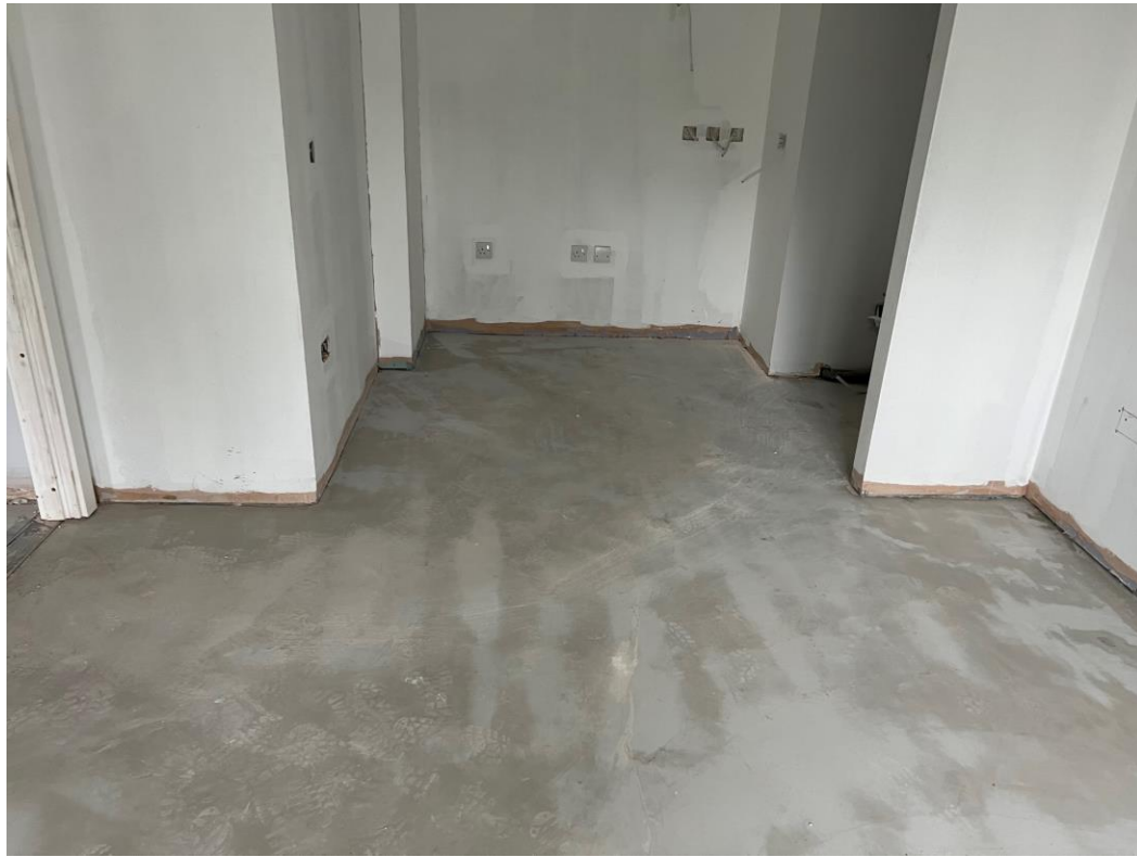
Level 2 – latex screed floors
