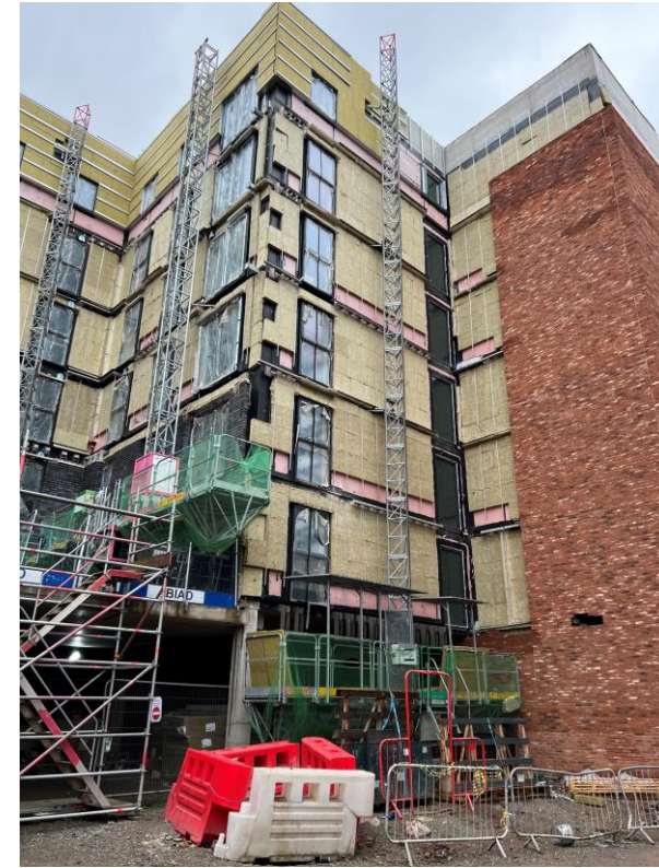
Block B wall insulation and brickwork
