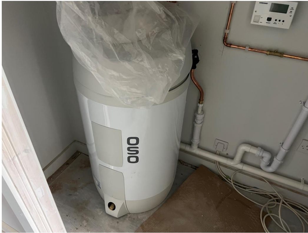
Level 5 – 2 nd fix mechanical installation
