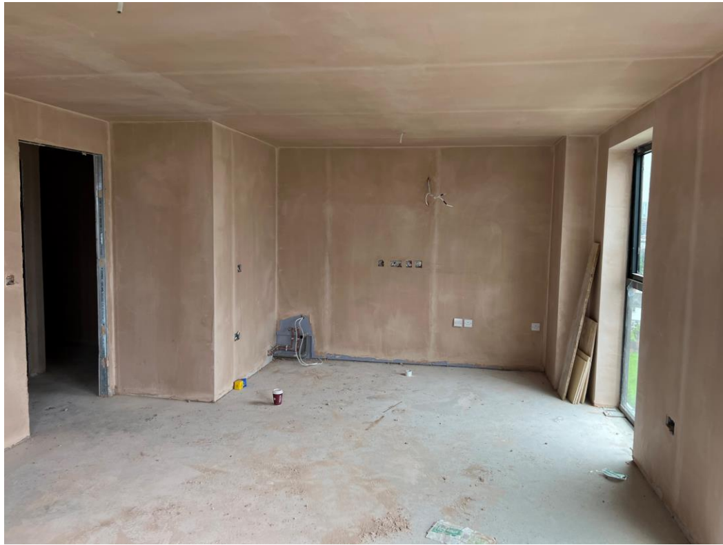
Level 8 – walls and ceilings plastered
