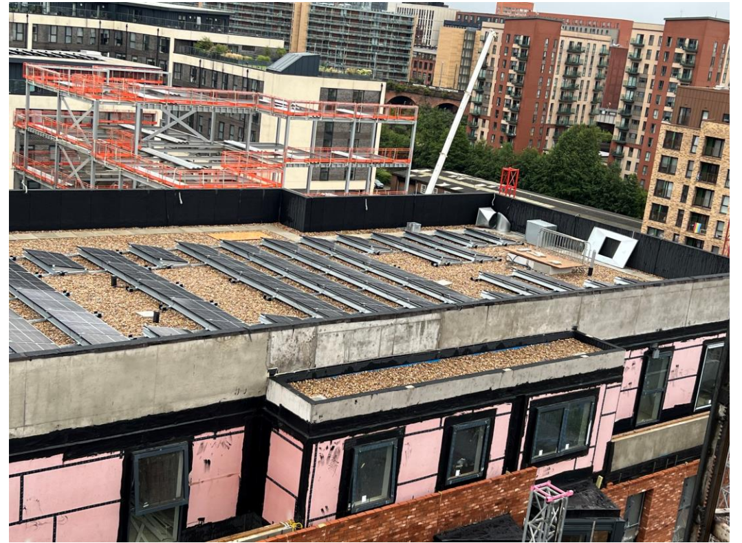
Block B inverted main roof system complete
