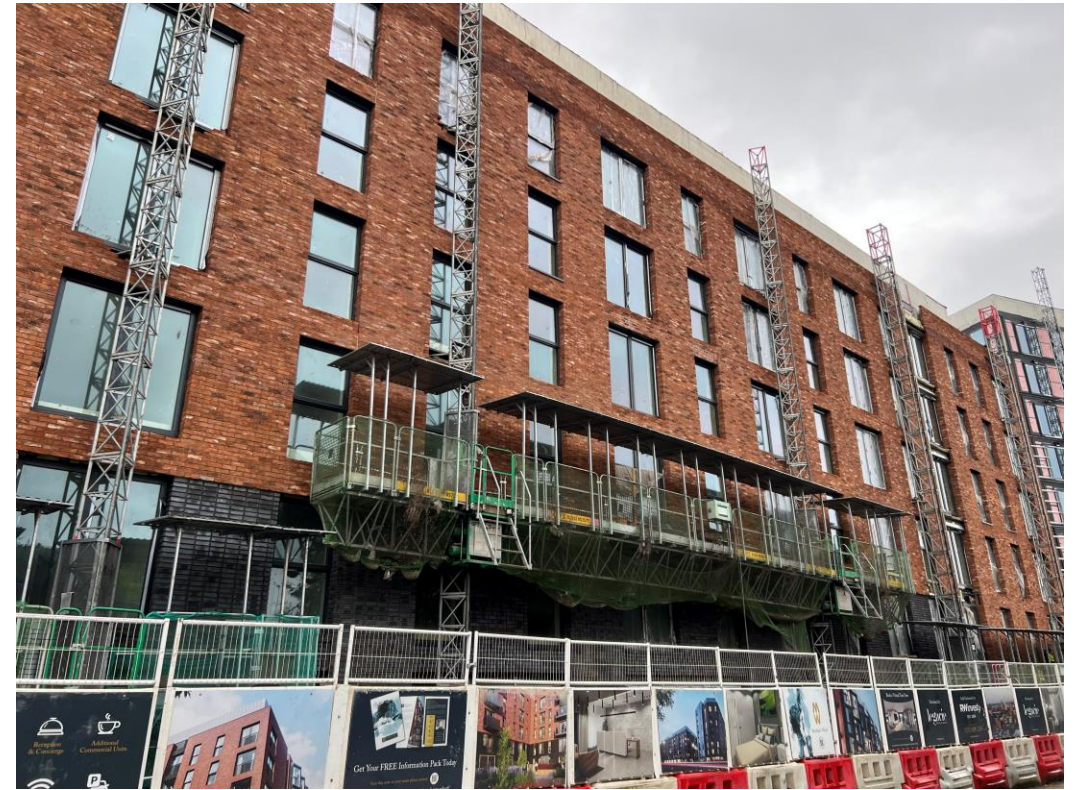
Ordsall Lane site view
