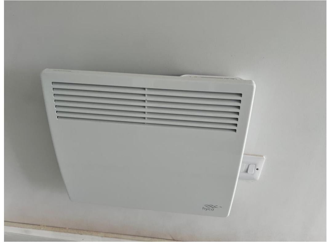
Level 5 – 2 nd fix mechanical installation
