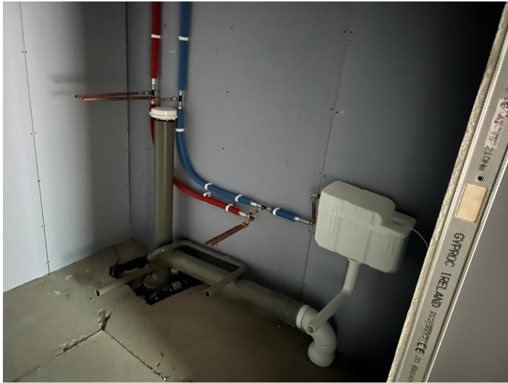
Ground Level – Apartments formed
