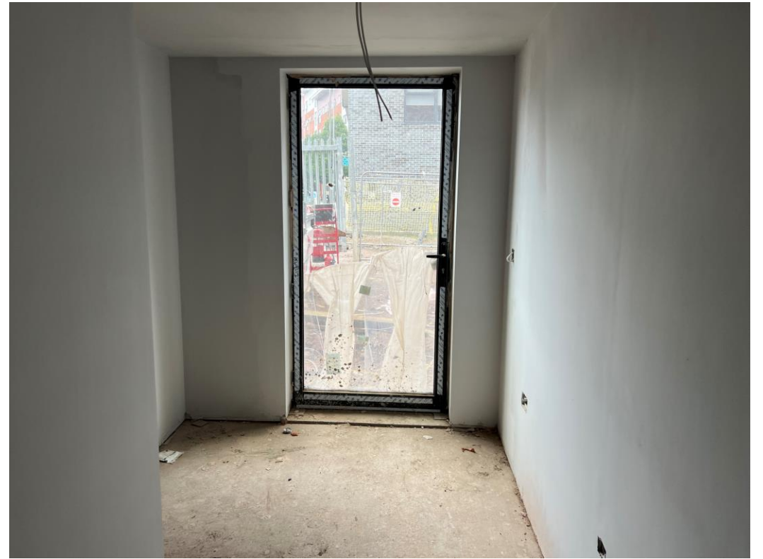
Ground Level 1 – Apartments formed
