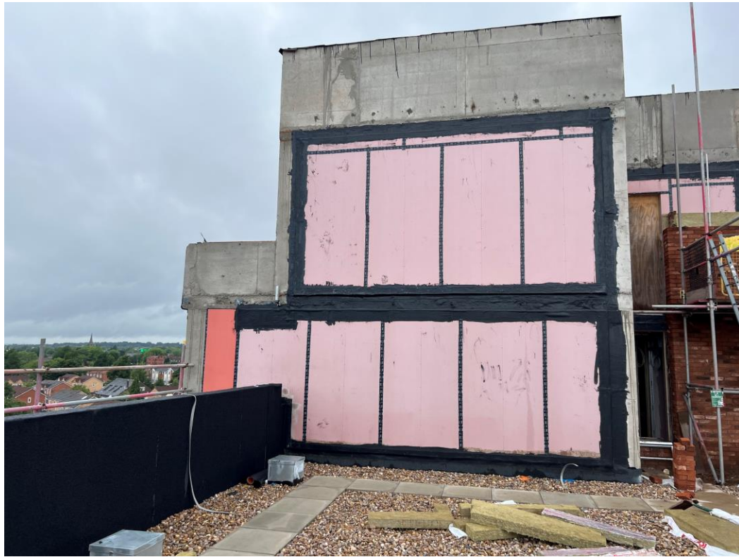
Block A wall insulation and brickwork
