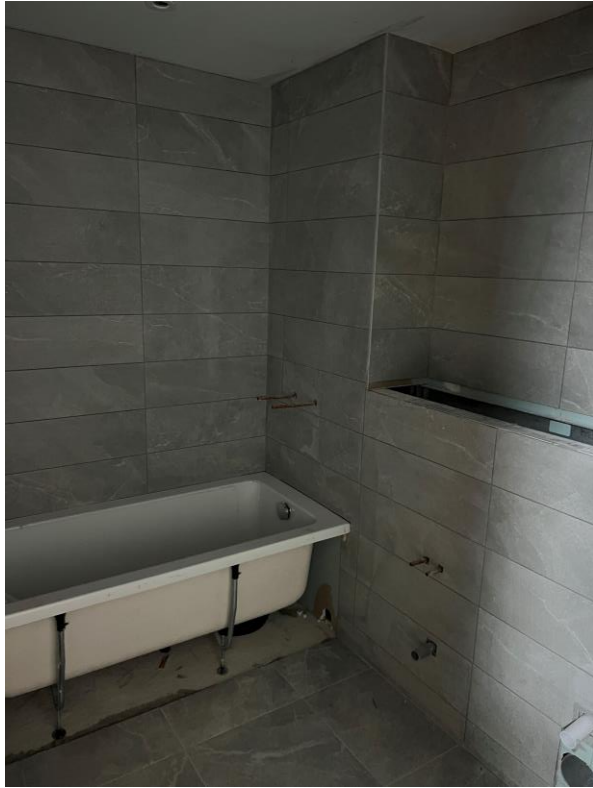
Level 6 – sanitary installation
