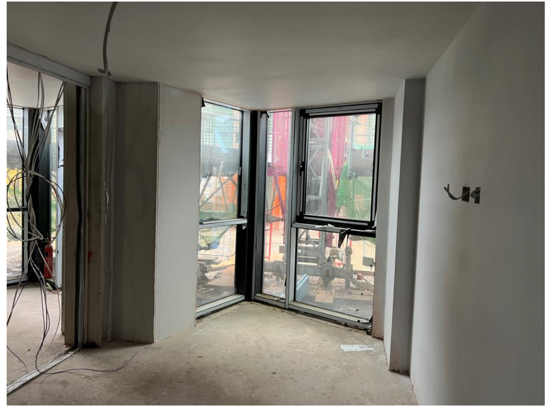
Ground Level 1 – Apartments formed
