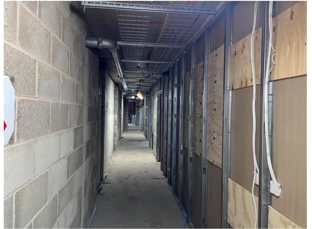
Ground Level – Apartments formed
