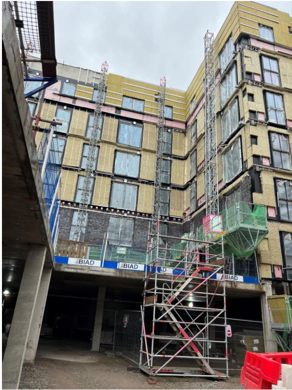
Block B wall insulation and brickwork
