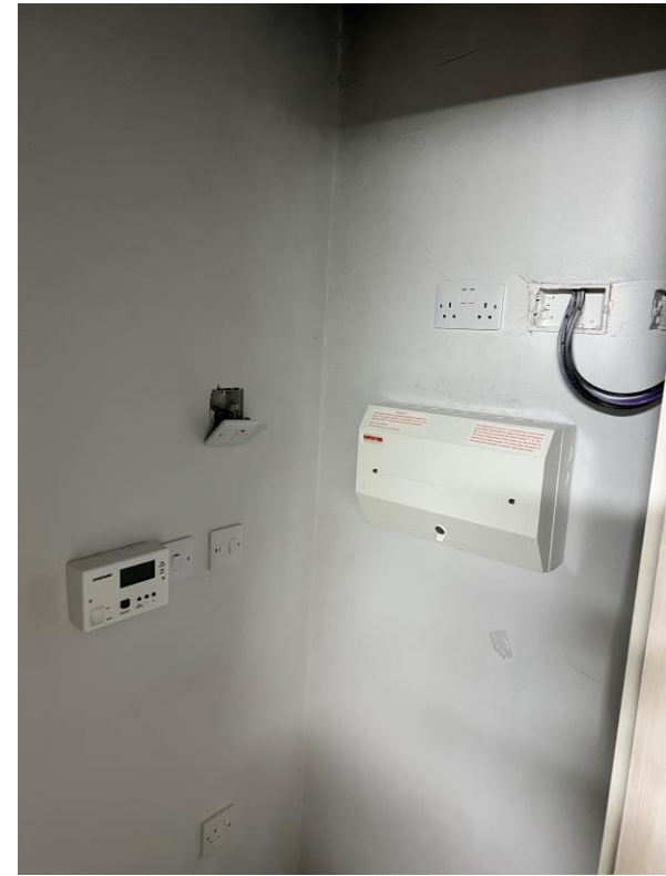
Level 6 – 2 nd fix electrical
