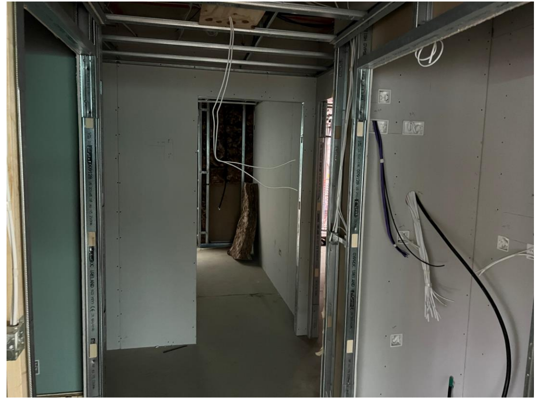
Ground Level – Apartments formed
