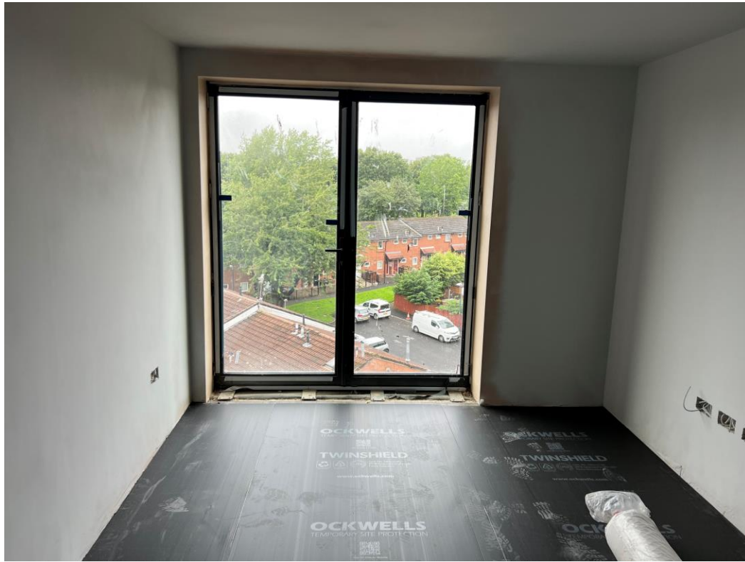
Level 5 – Laminate floor covering installed
