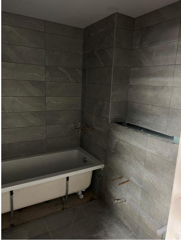
Level 5 – wall and floor tiling
