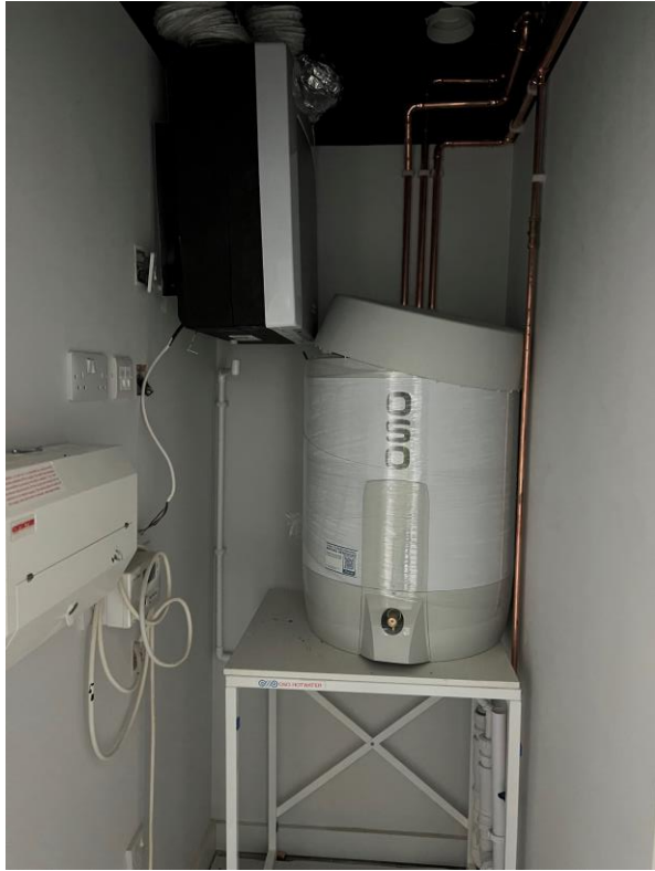
Level 2 – 2 nd fix mechanical
