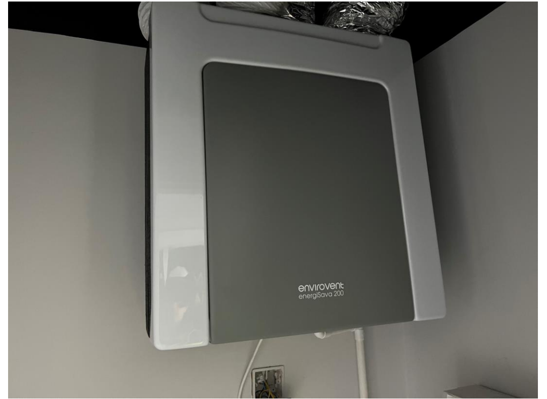
Level 5 – 2 nd fix mechanical installation
