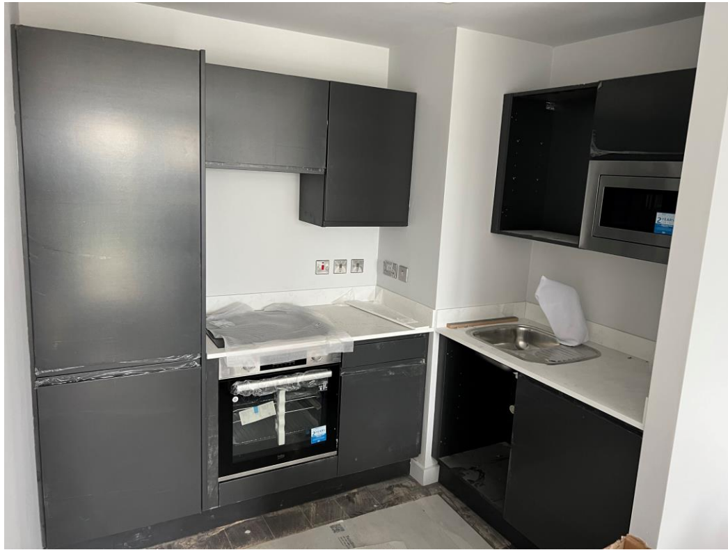
Level 4 – Kitchen units installed
