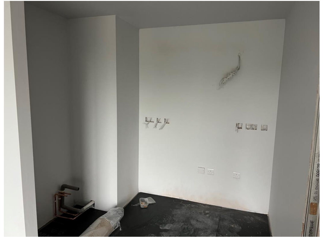
Level 5 – Kitchen prepared for units
