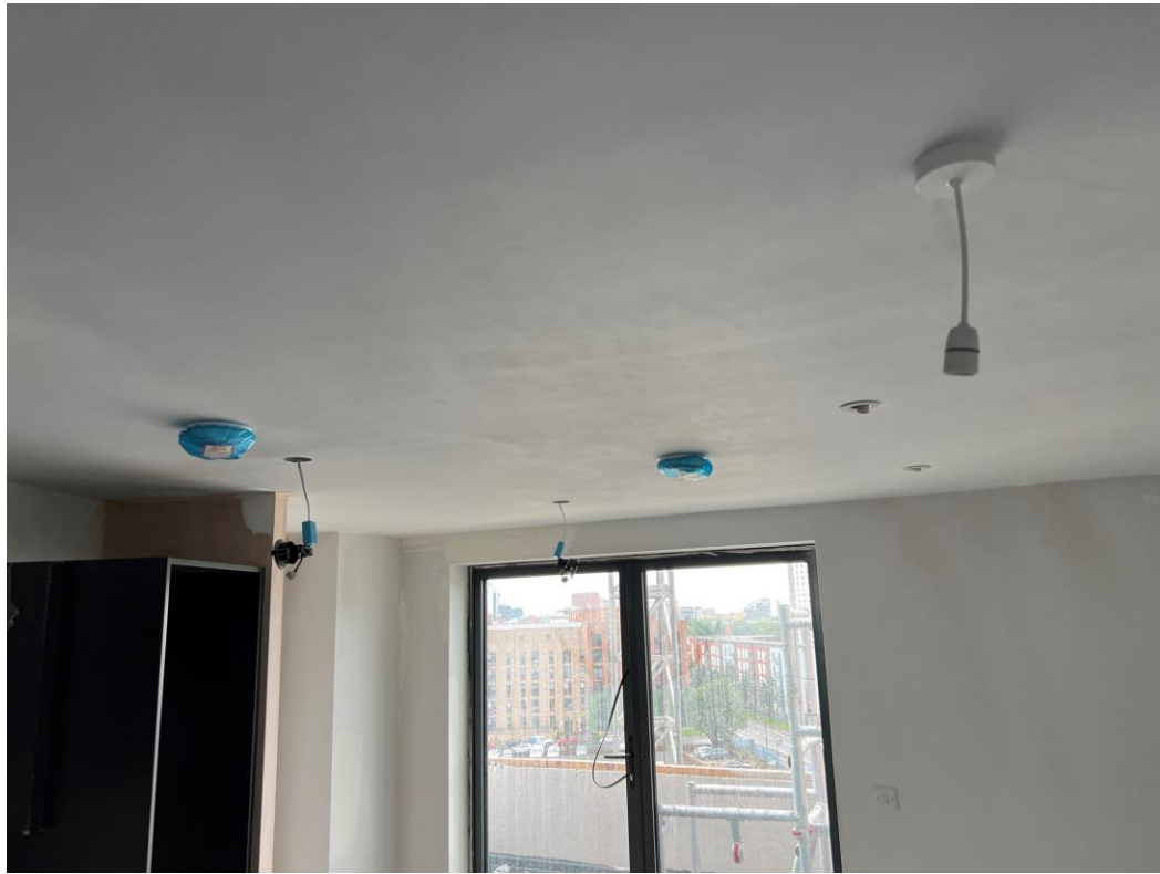
Level 6 – 2 nd fix electrical
