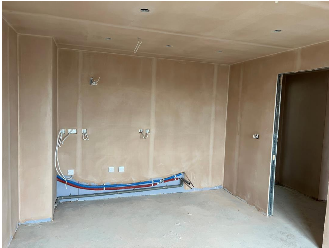
Level 8 – walls and ceilings plastered
