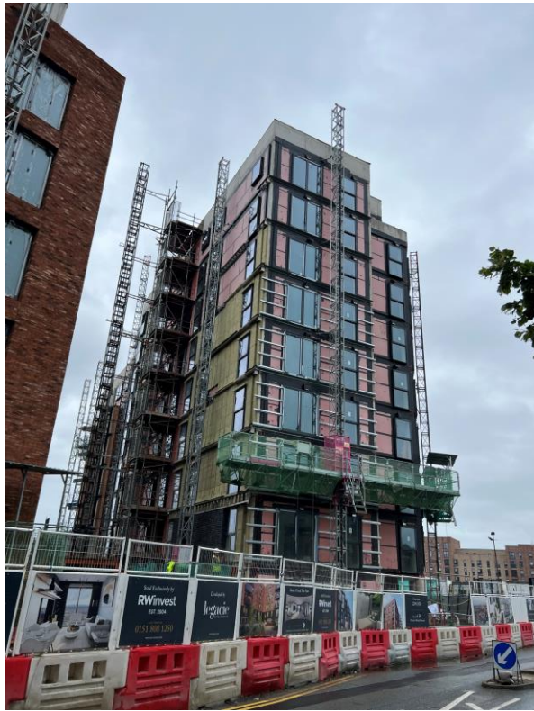
Ordsall Lane site view
