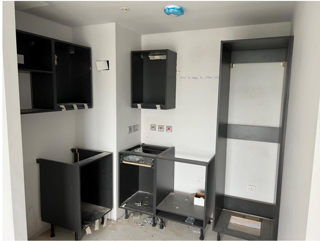
Level 7 – Kitchen units installed
