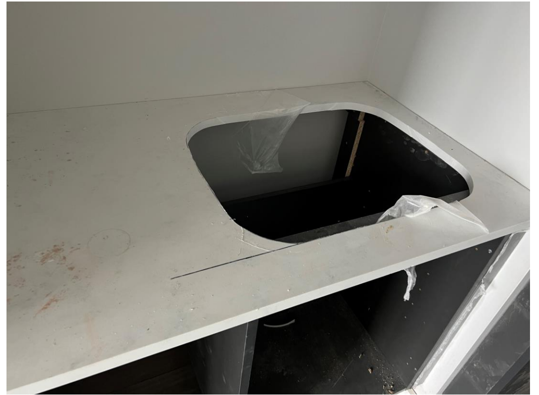
Level 6 – Kitchen units installed
