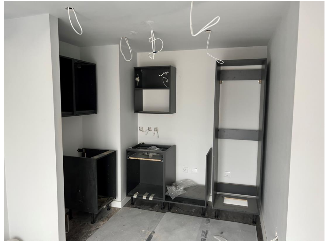
Level 6 – Kitchen units installed
