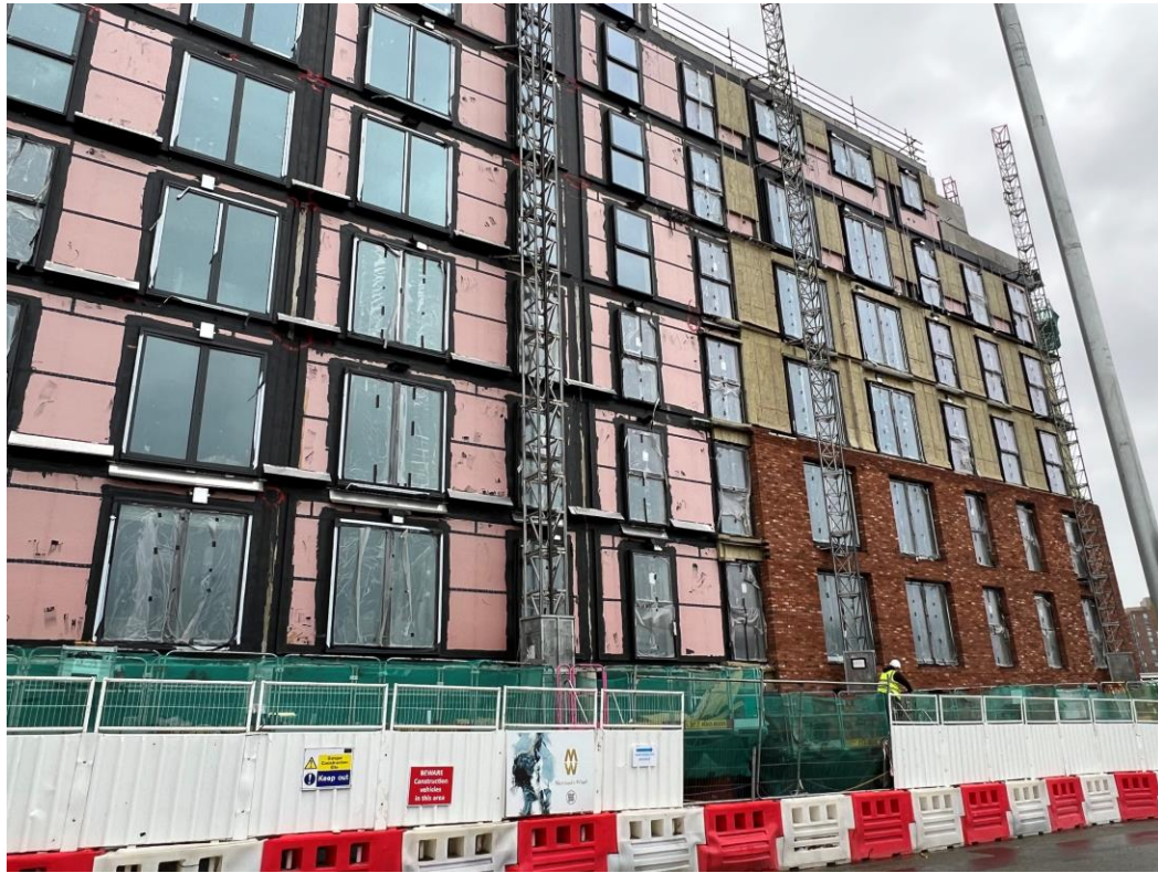
Ordsall Lane site view
