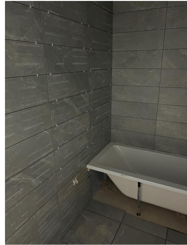
Level 5 – wall and floor tiling
