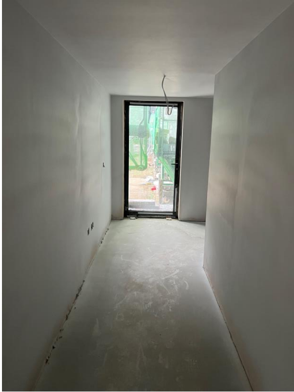
Level 1 – latex screed floors
