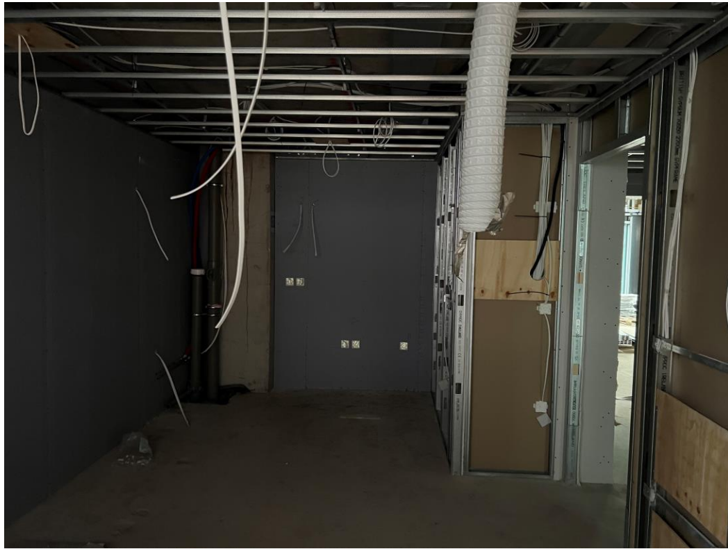
Ground Level – Apartments formed
