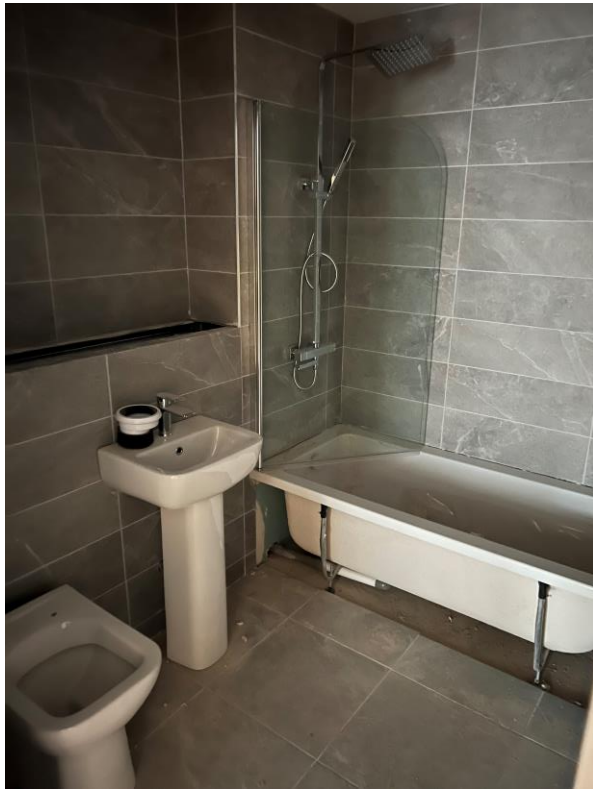
Level 3 – Bathroom fittings installed
