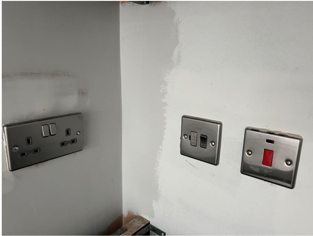
Level 2 – 2 nd fix electrical sockets
