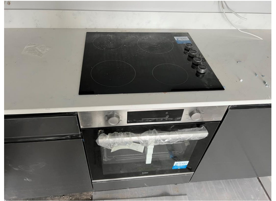
Level 4 – Kitchen units installed
