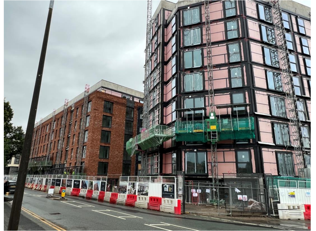
Ordsall Lane site view
