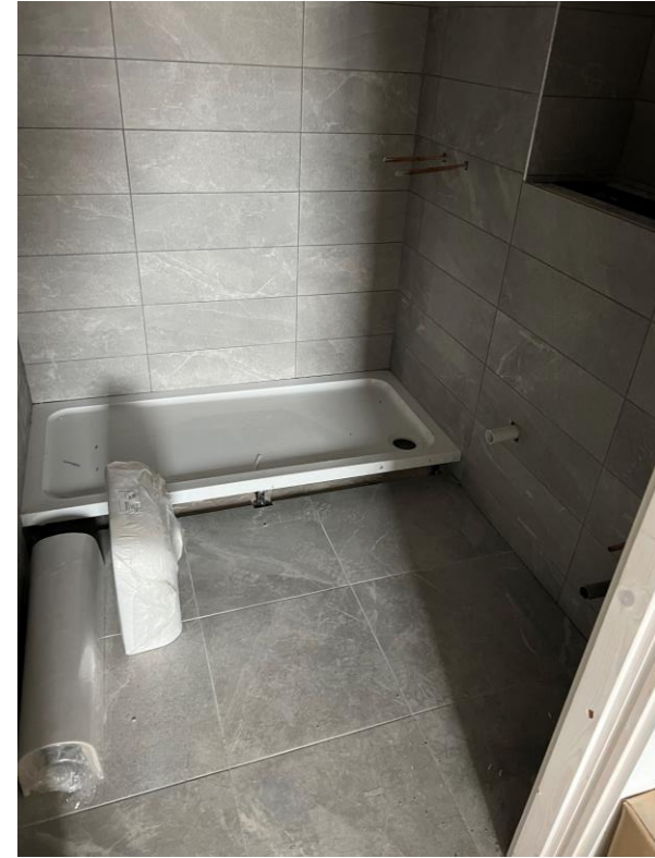
Level 6 – sanitary installation
