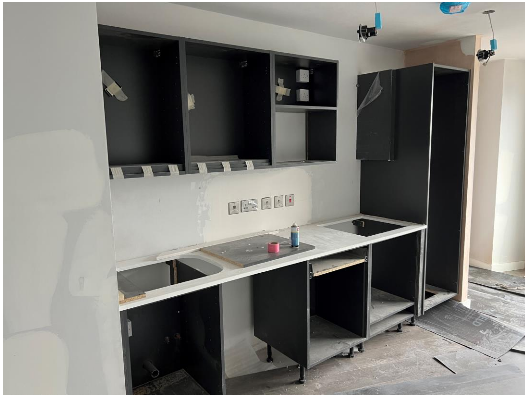
Level 6 – Kitchen units installed
