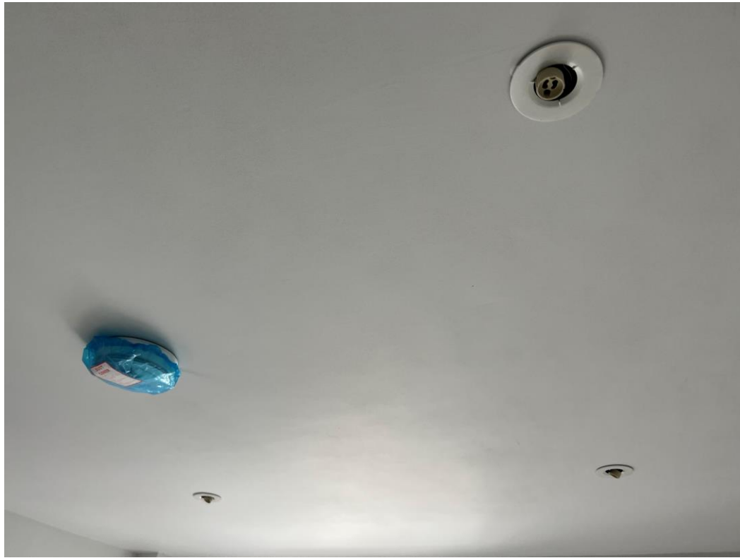
Level 7 – 2 nd fix electrical
