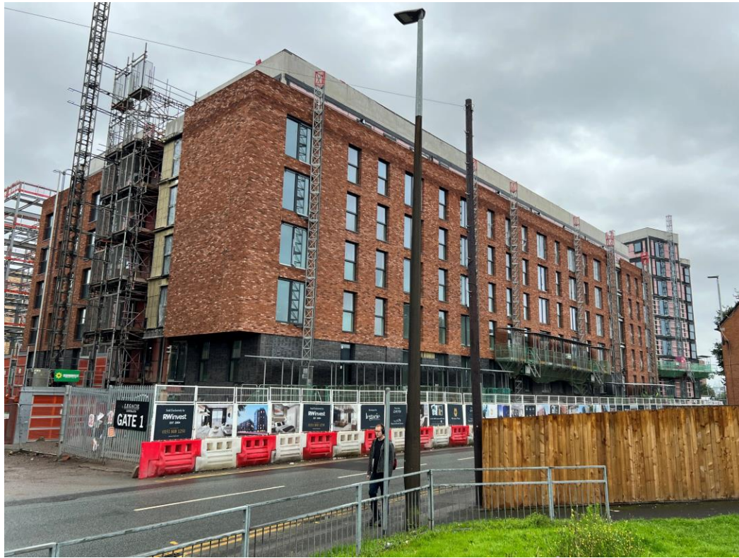
Ordsall Lane site view
