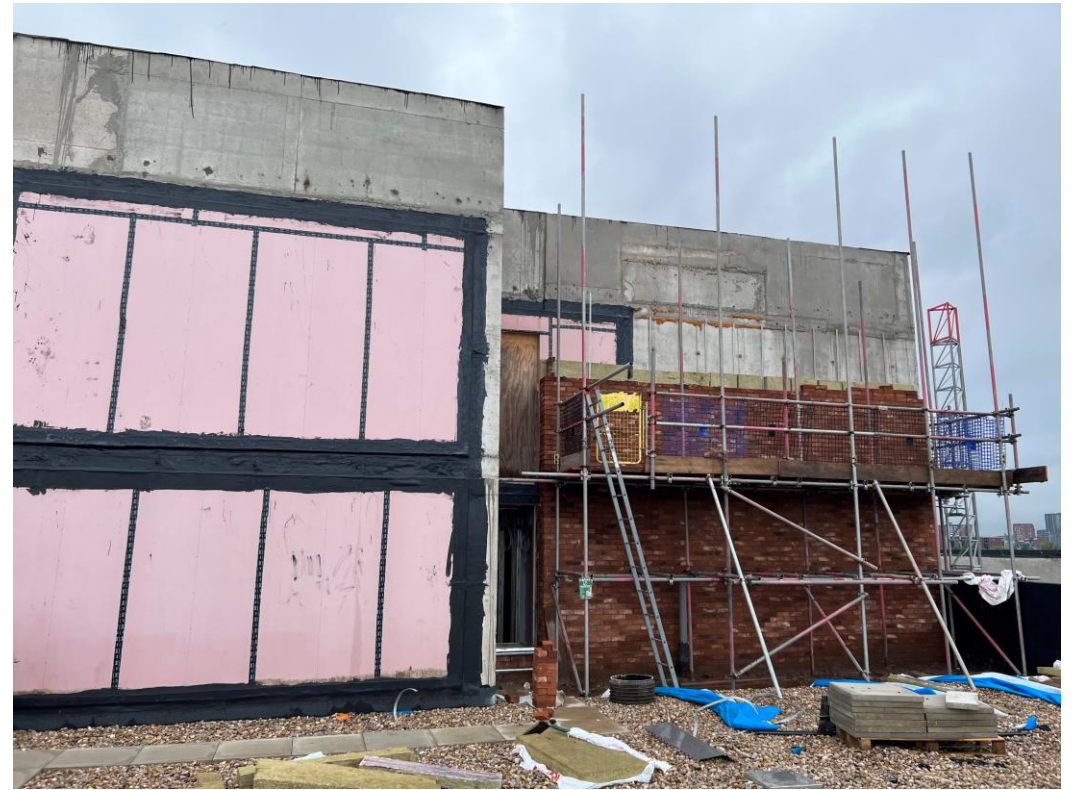
Block A wall insulation and brickwork
