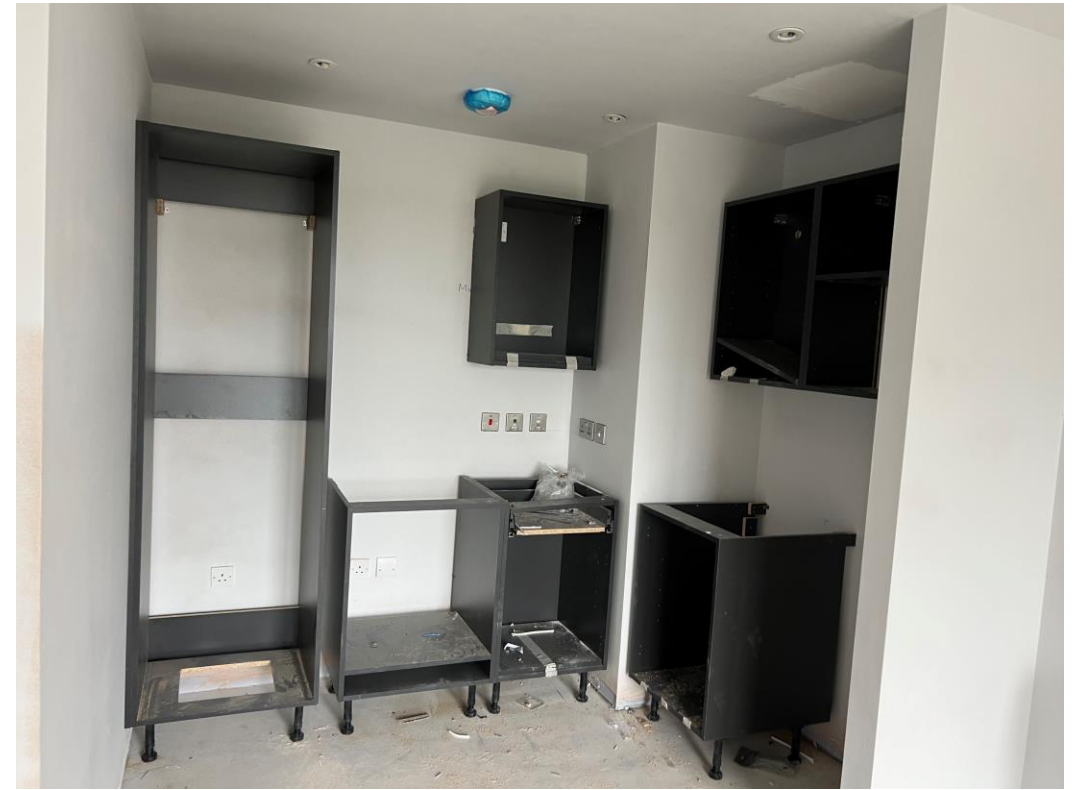
Level 7 – Kitchen units installed
