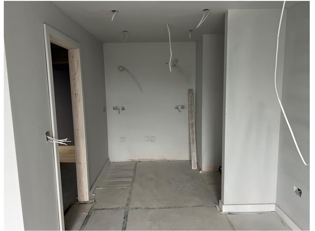
Level 4 – doorcasings, skirting and architrave
