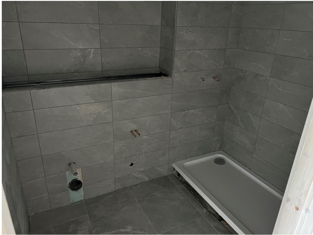
Level 6 – wall and floor tiling
