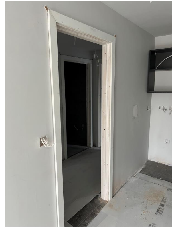
Level 6 – doorcasings, skirting and architrave
