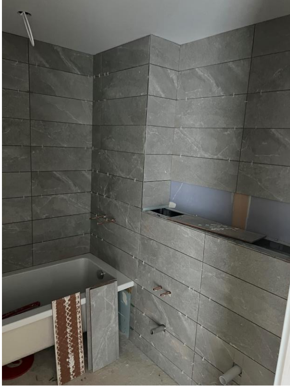
Level 2 – wall and floor tiling
