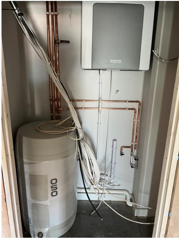
Level 3 – 2 nd fix mechanical
