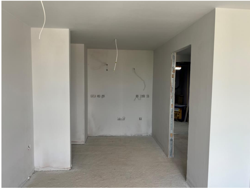
Level 6 – Apartment decoration walls and ceiling
