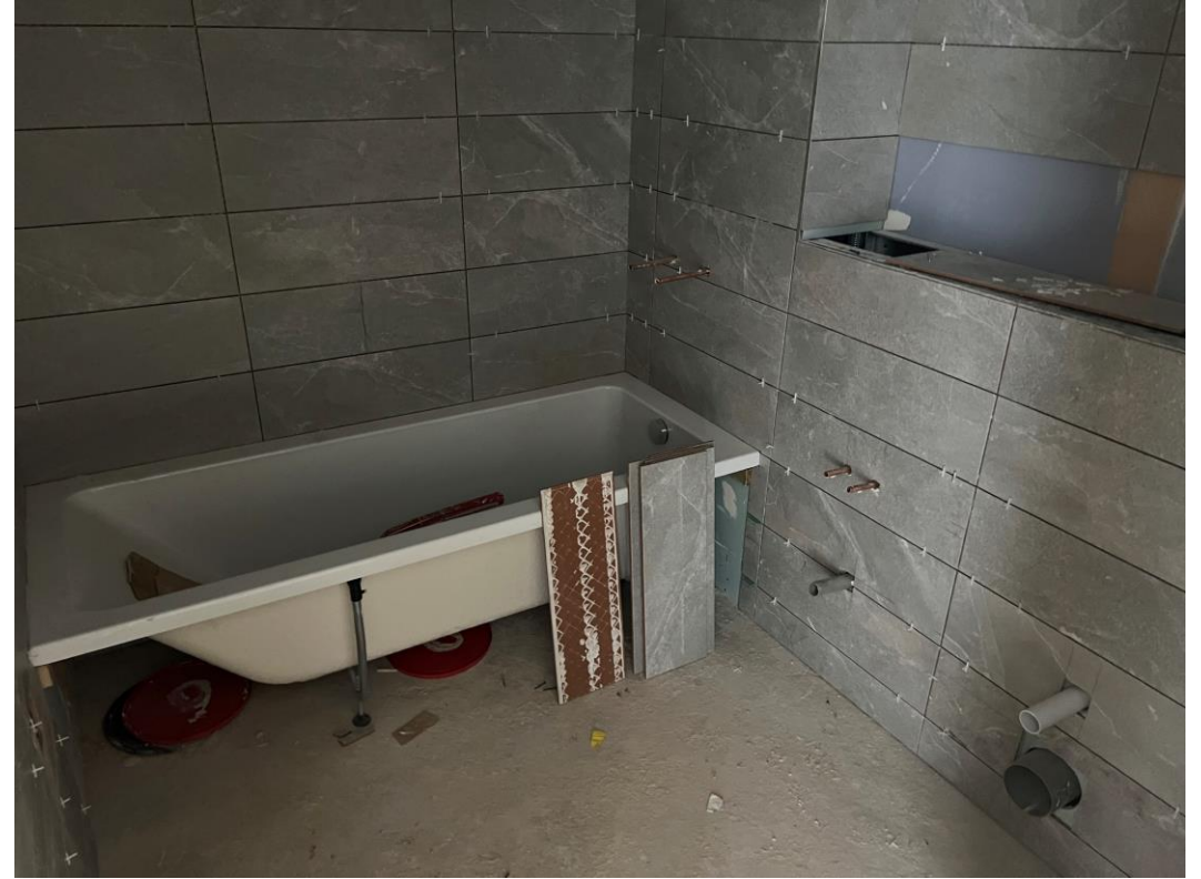
Level 2 – wall and floor tiling
