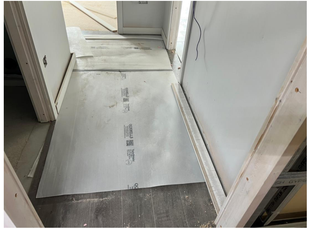
Level 4 – Laminate flooring installed
