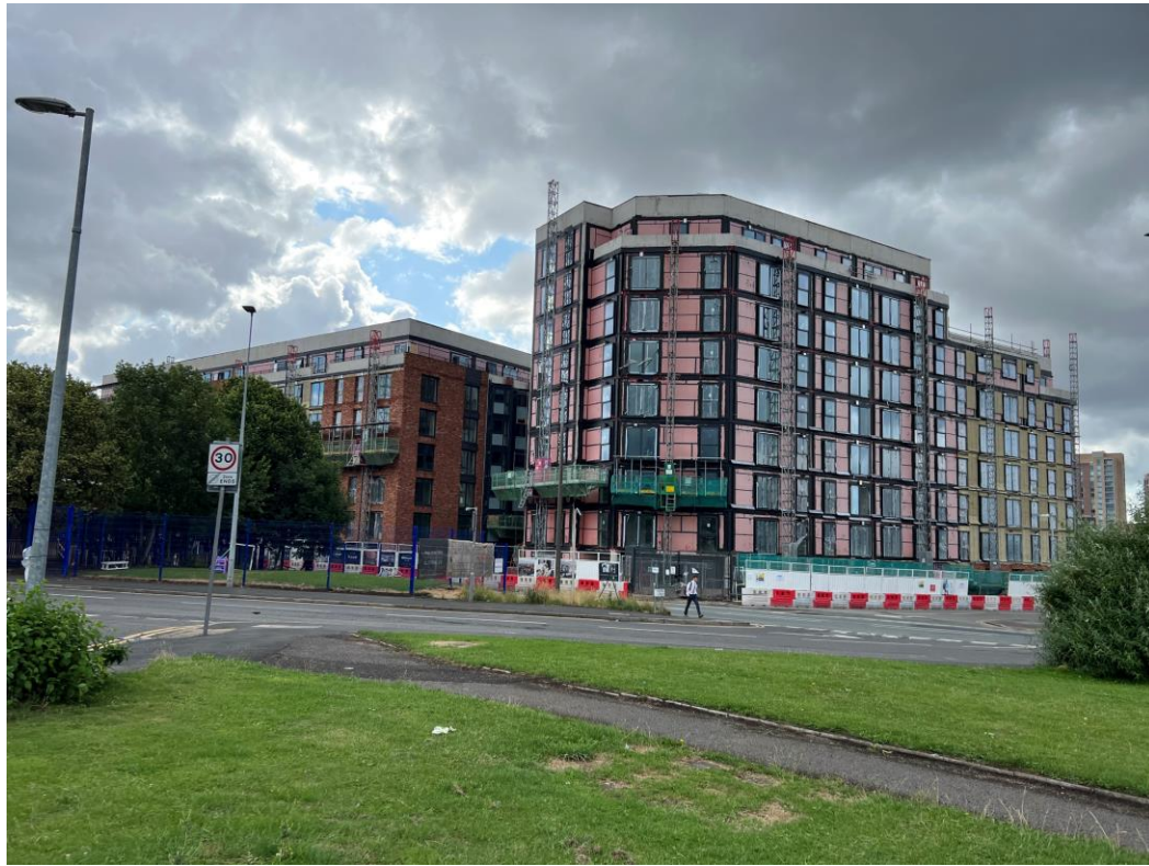
Ordsall Lane site view
