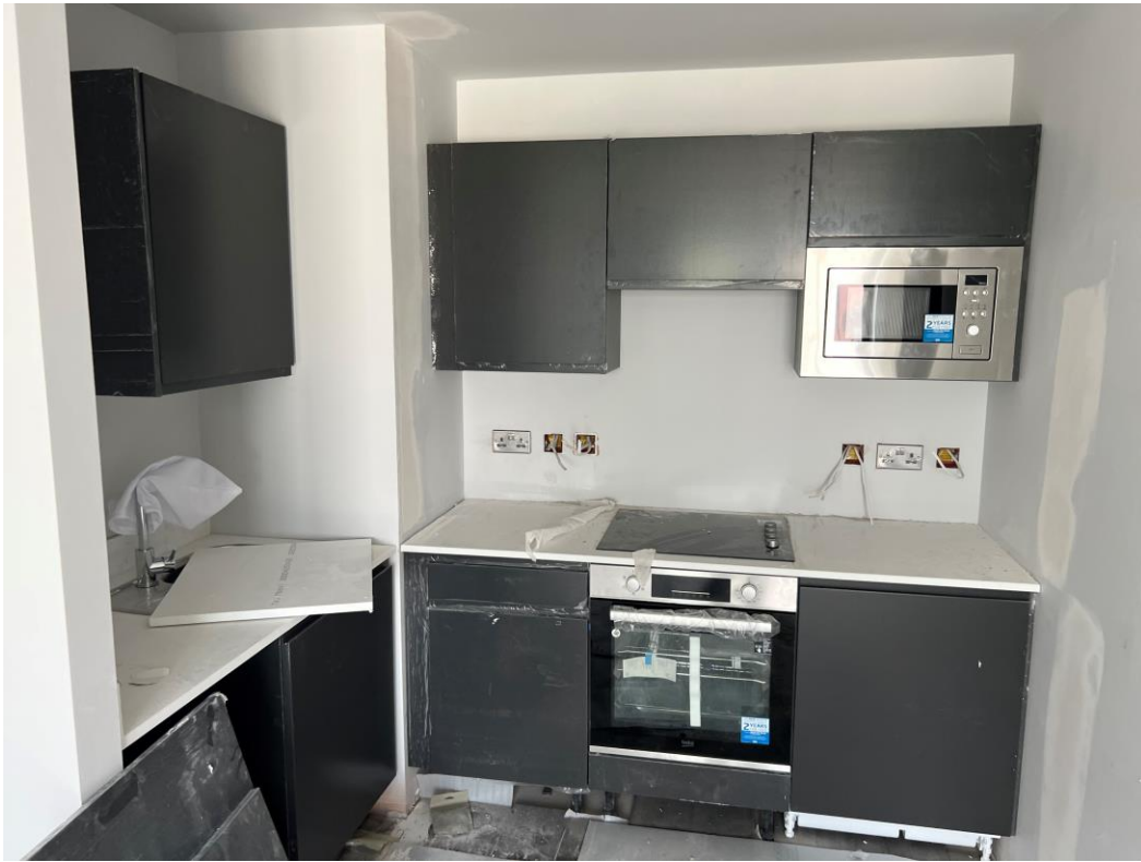
Level 3 – Kitchen units installed
