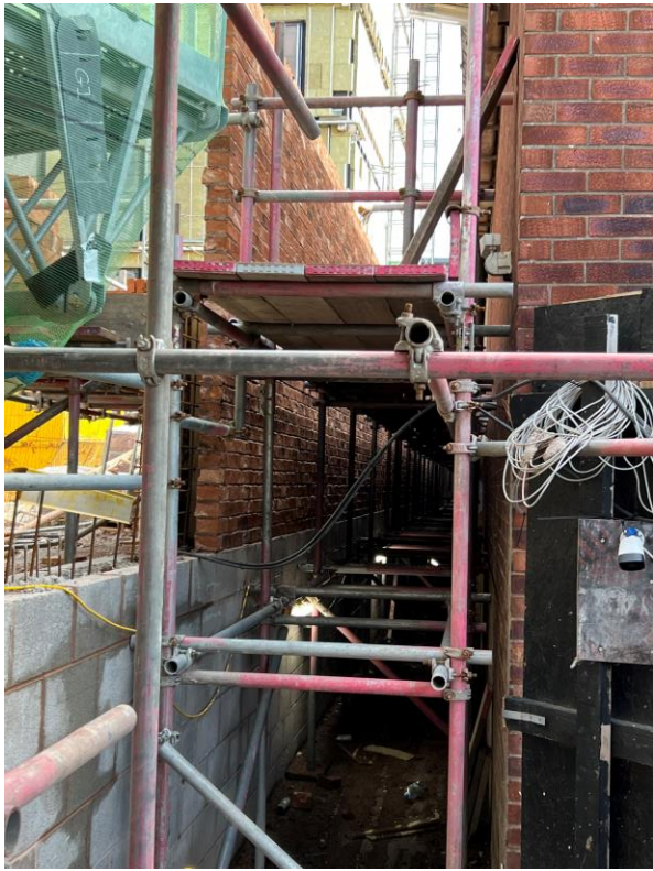
Block A wall insulation and brickwork
