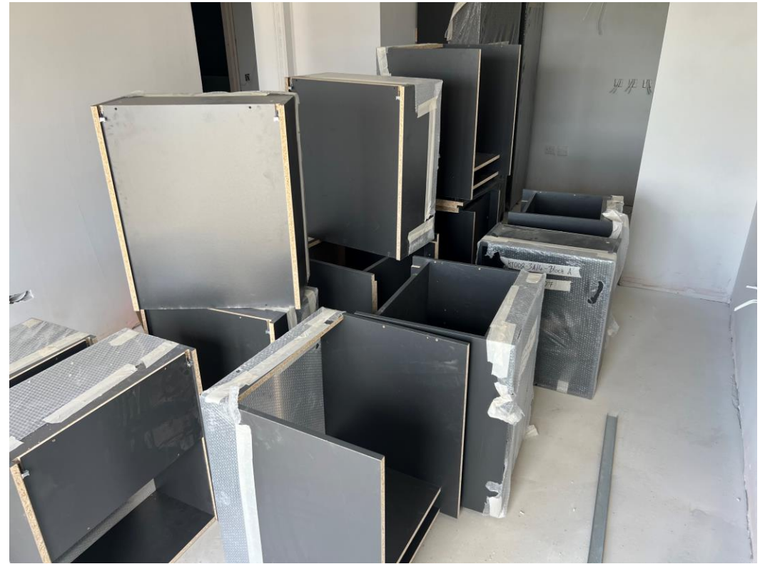
Level 4 – Kitchen units installed
