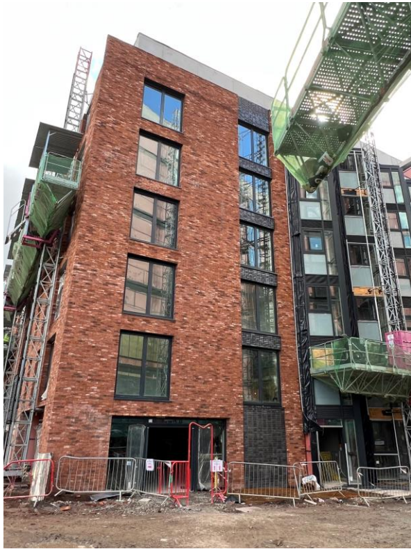
Block B Curtain walling and brickwork
