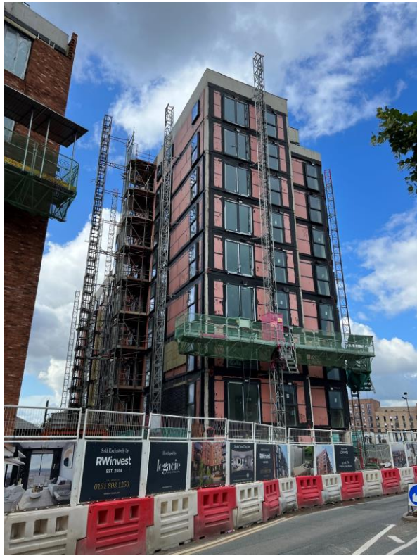
Ordsall Lane site view
