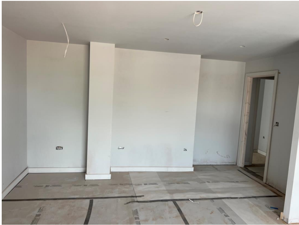
Level 4 – doorcasings, skirting and architrave
