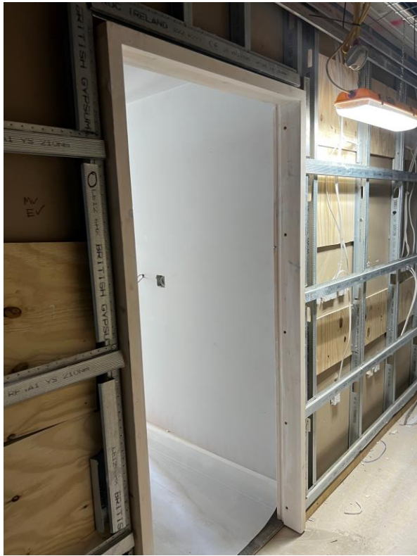
Level 4 – doorframes installed
