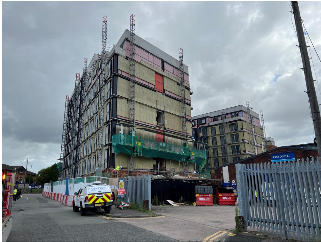
Worrall Street site view
