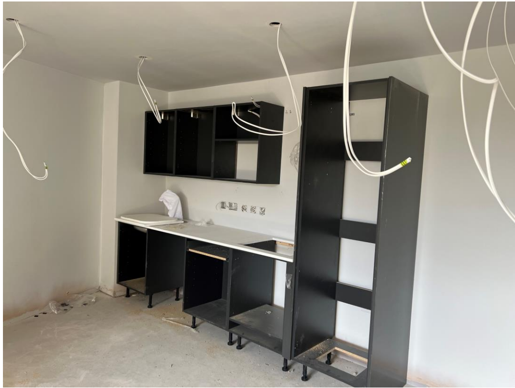
Level 4 – Kitchen units installed
