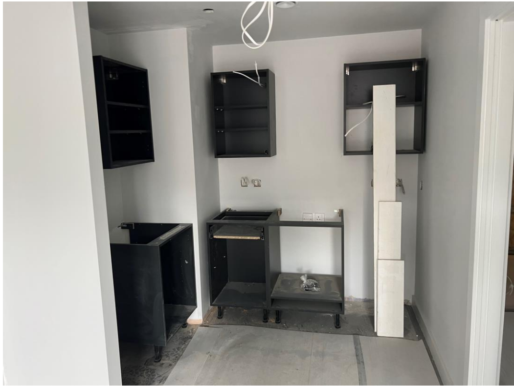
Level 1 – Kitchen units installed
