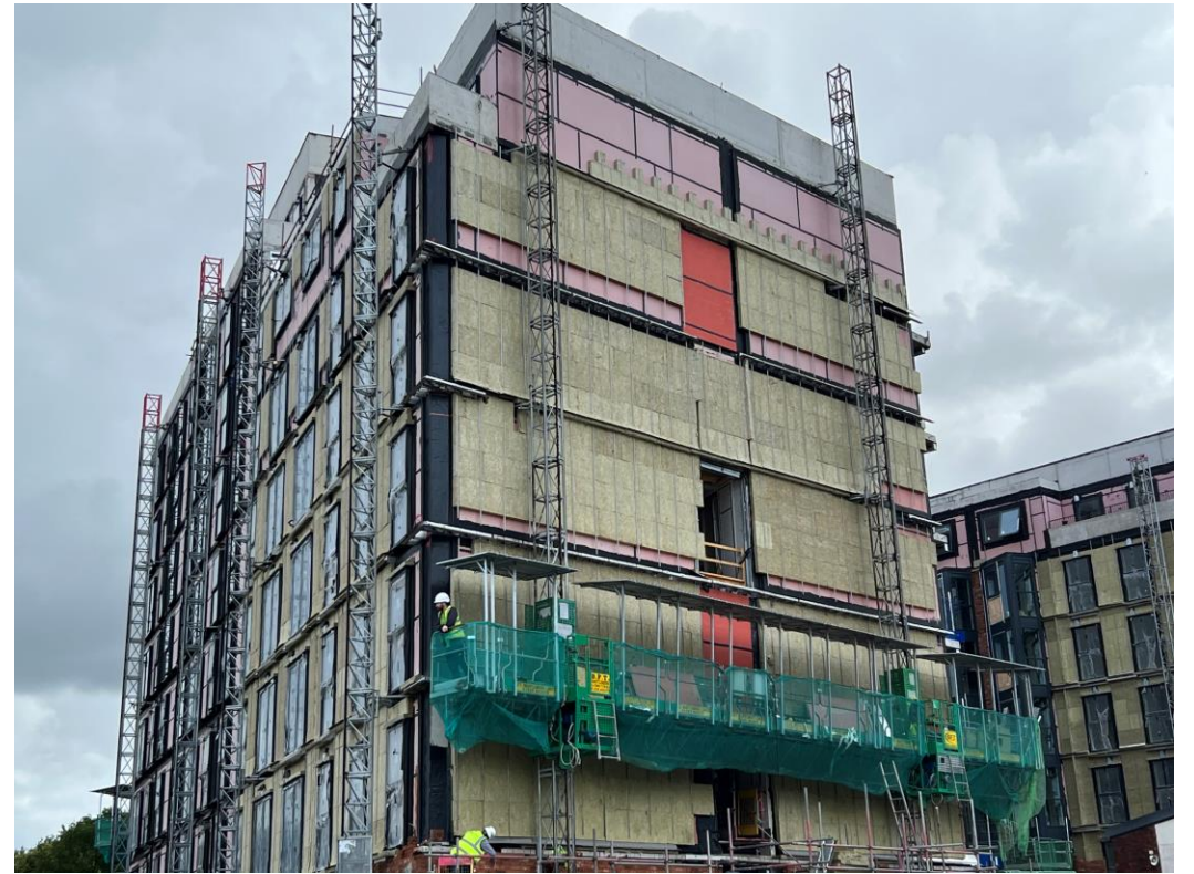
Worrall Street site view
