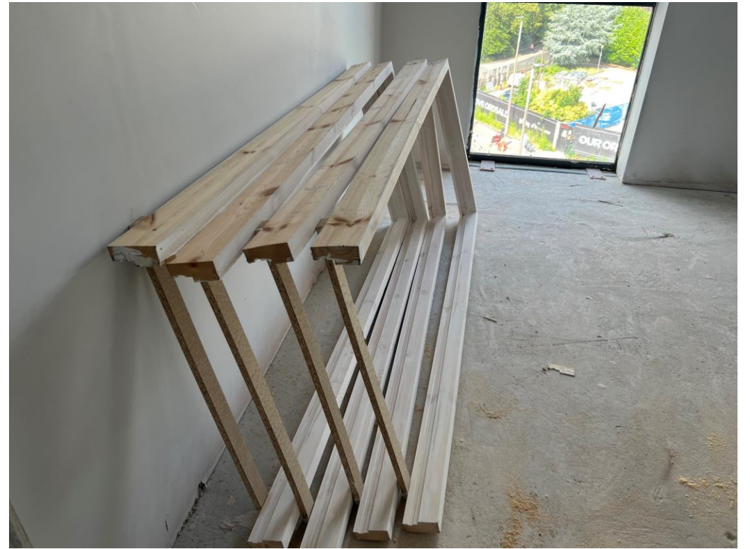
Level 5 – doorframes loaded ready for installation
