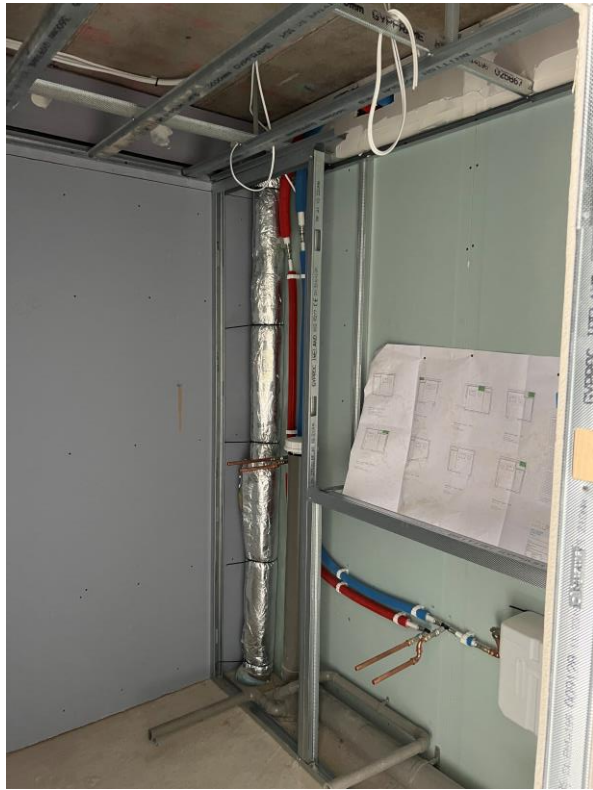
Level 8 – first fix plumbing
