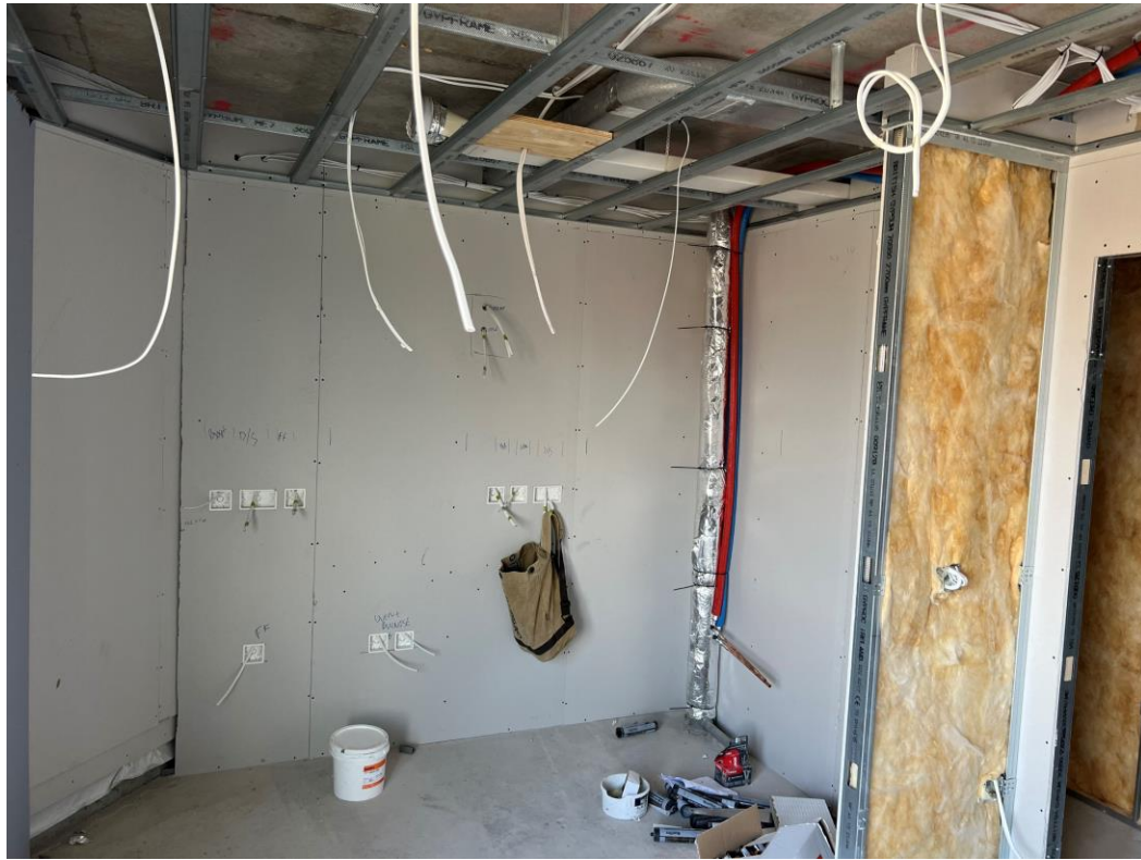
Level 8 – apartment walls and ceilings formed
