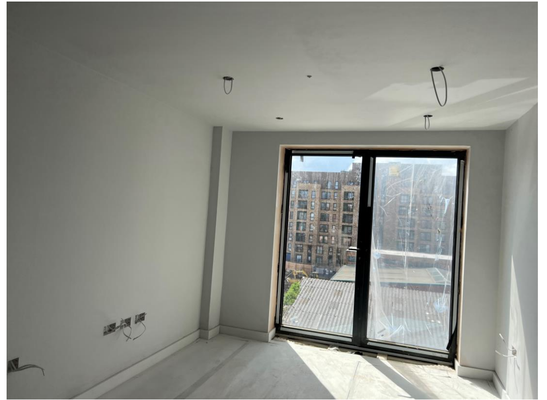
Level 4 – doorcasings, skirting and architrave
