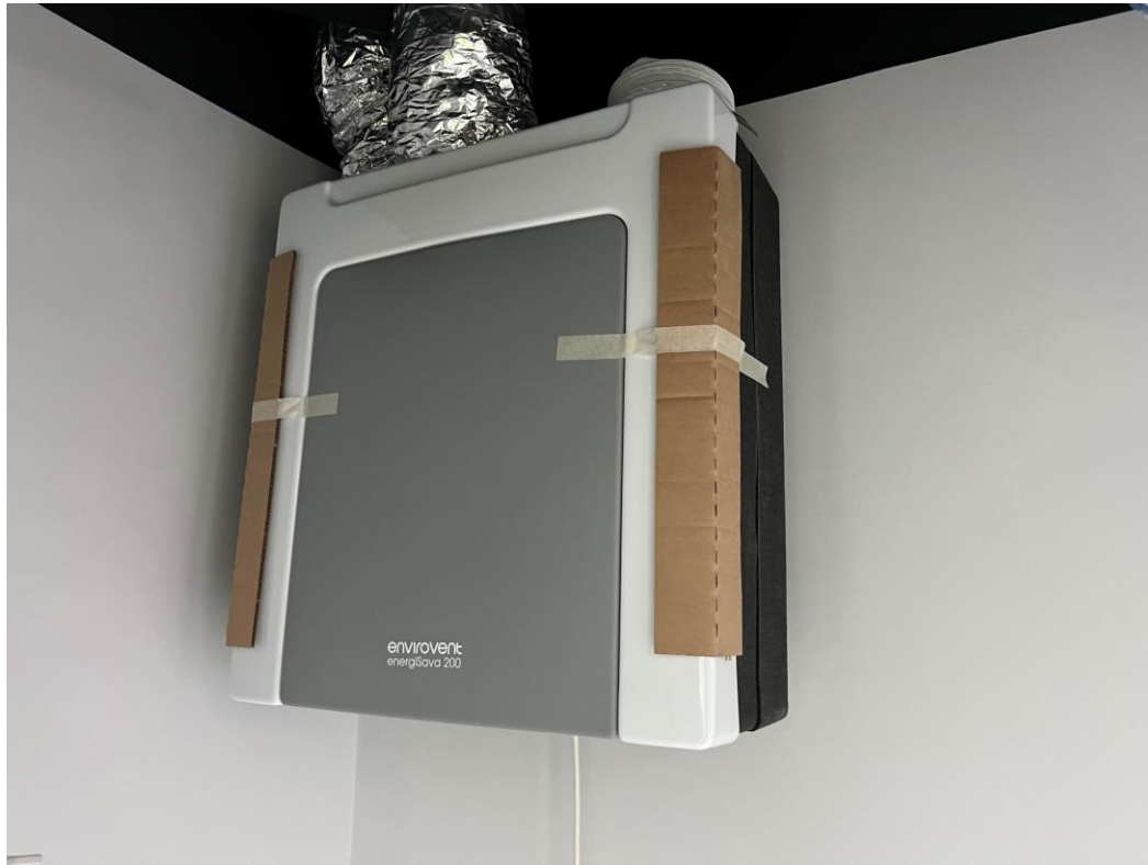
Level 5 – 2 nd fix mechanical installation
