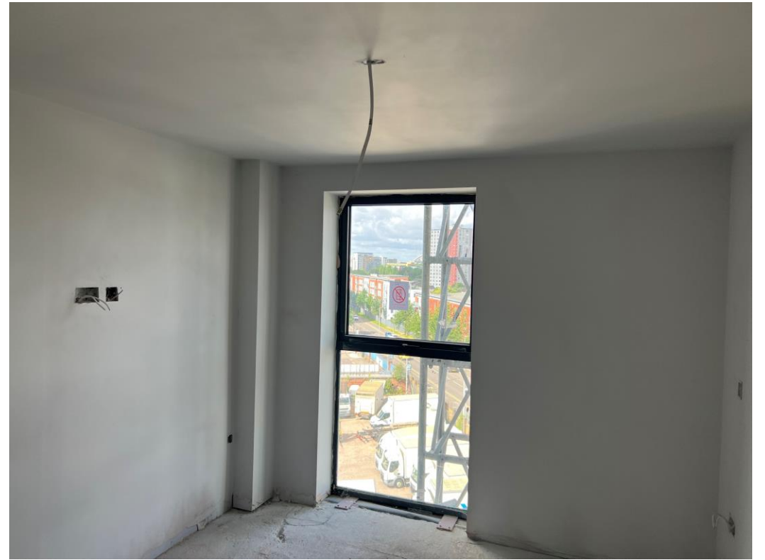
Level 6 – Apartment decoration walls and ceiling
