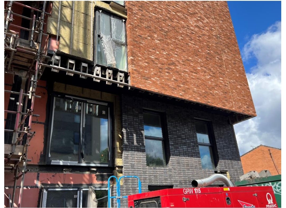
Block B wall insulation and brickwork
