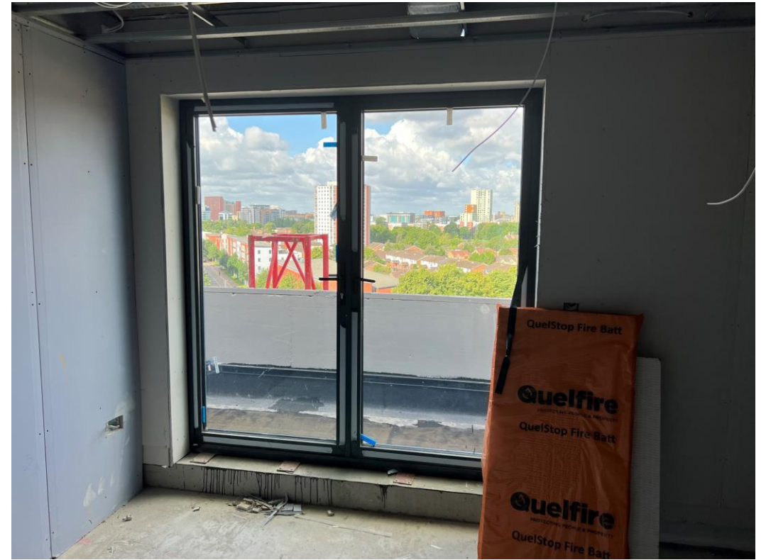
Level 8 – external walls insulated and plasterboarded
