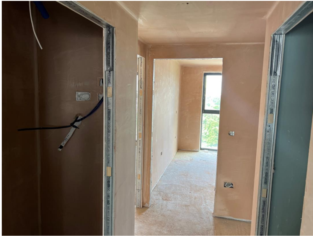
Level 7 – walls and ceilings plastered
