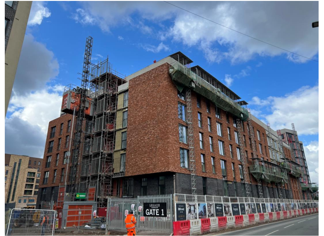
Ordsall Lane site view
