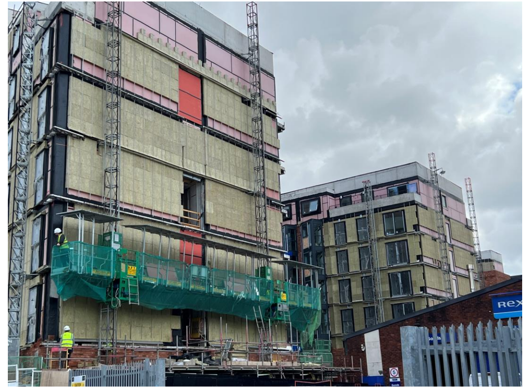
Worrall Street site view
