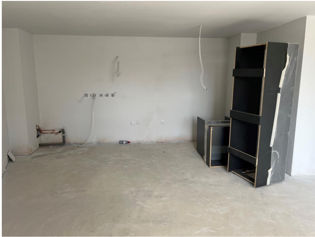
Level 5 – Kitchen units loaded ready for installation
