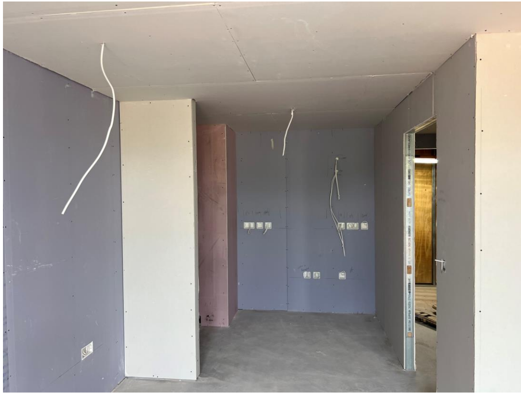
Level 5 – apartments prepared for plastering
