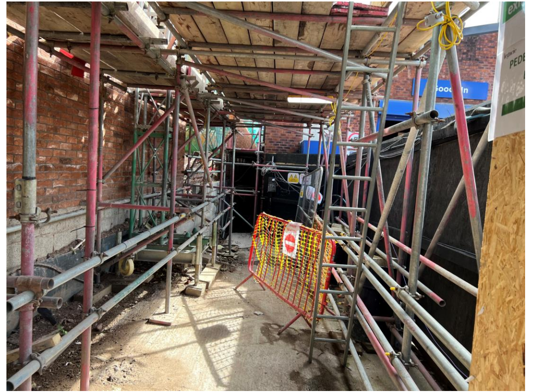
Block A wall insulation and brickwork
