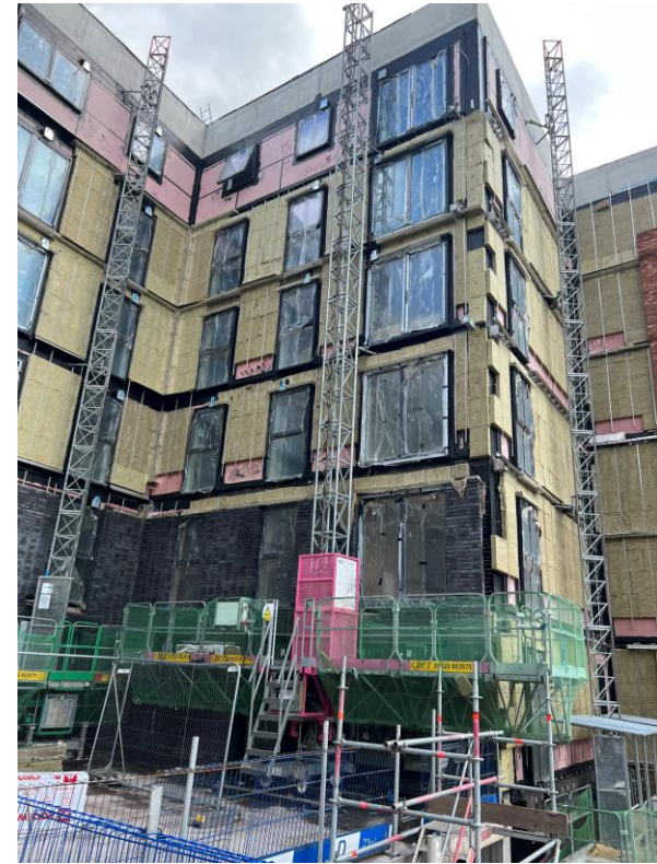
Block B wall insulation and brickwork
