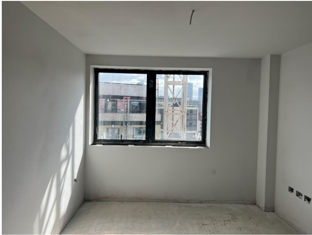
Level 6 – Apartment decoration walls and ceiling
