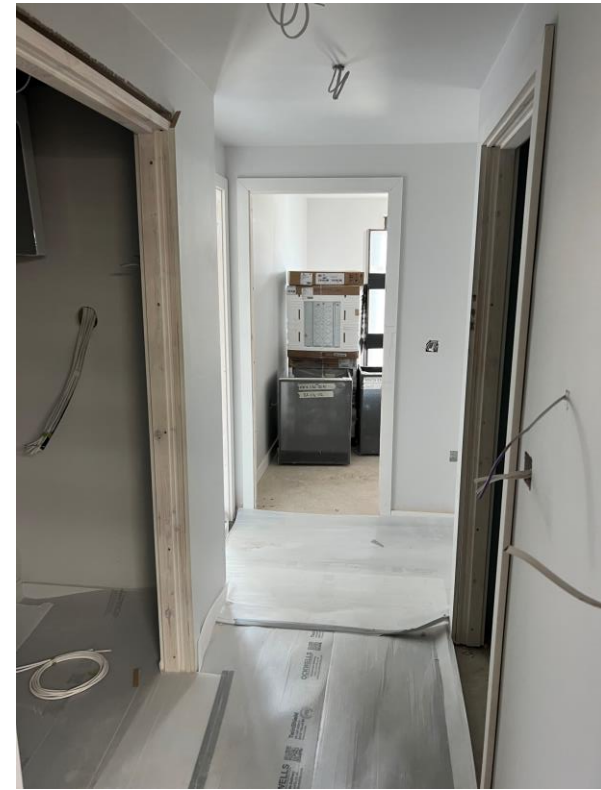
Level 4 – doorframes installed
