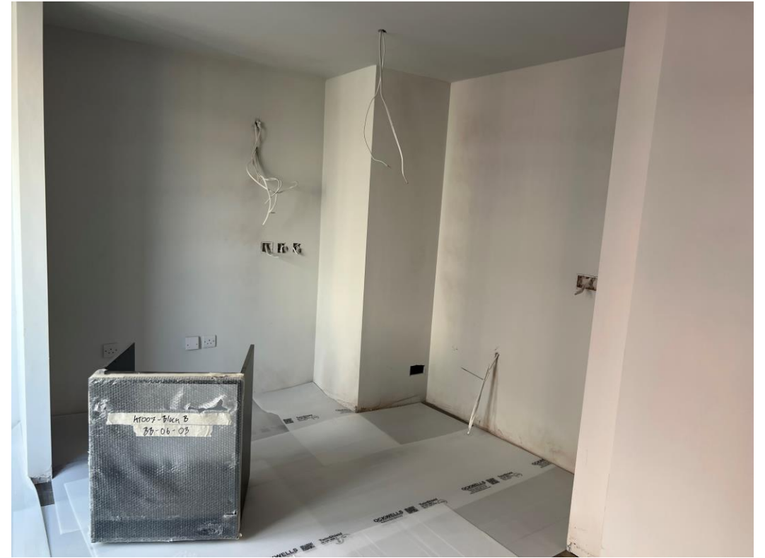
Level 6 – corridor and apartment walls formed
