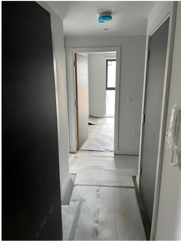
Level 1 – doors installed
