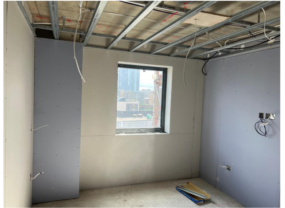
Level 8 – apartment walls and ceilings formed
