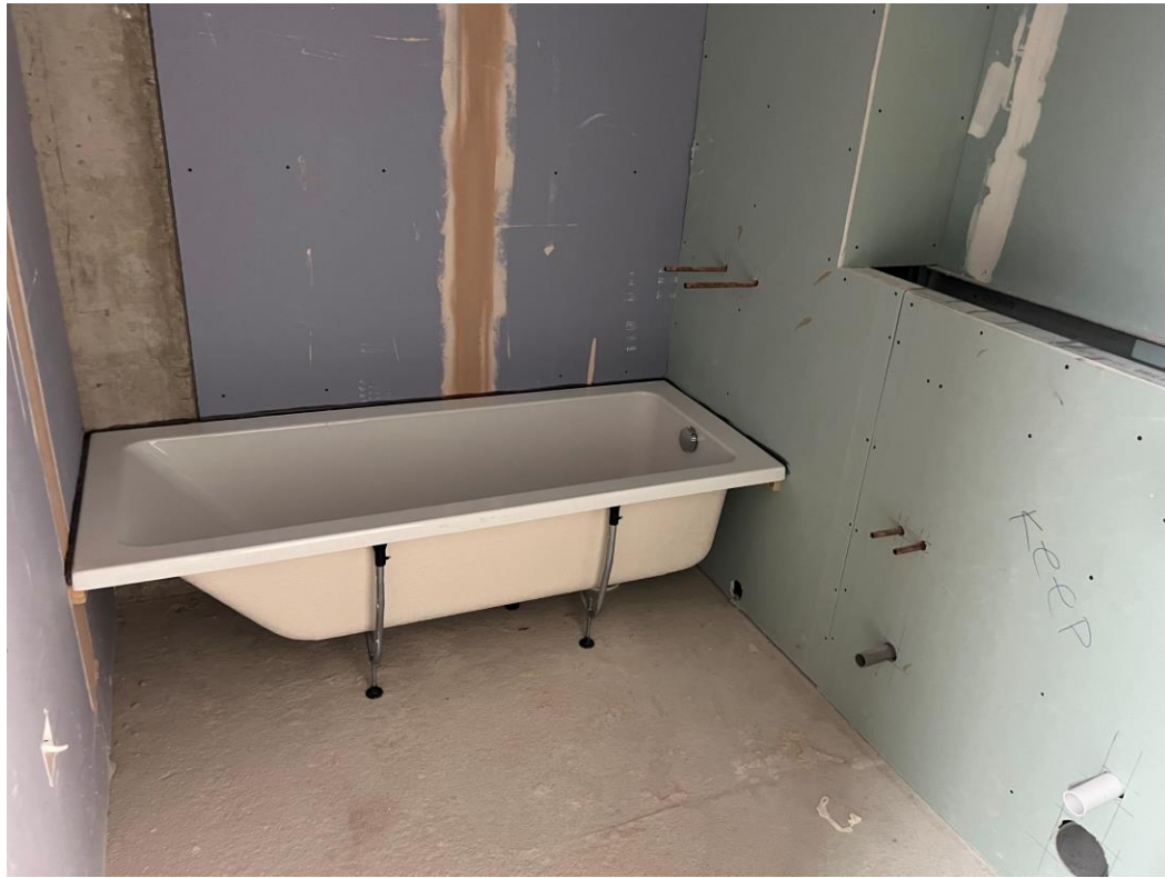
Level 6 – IPS formed & sanitary installation
