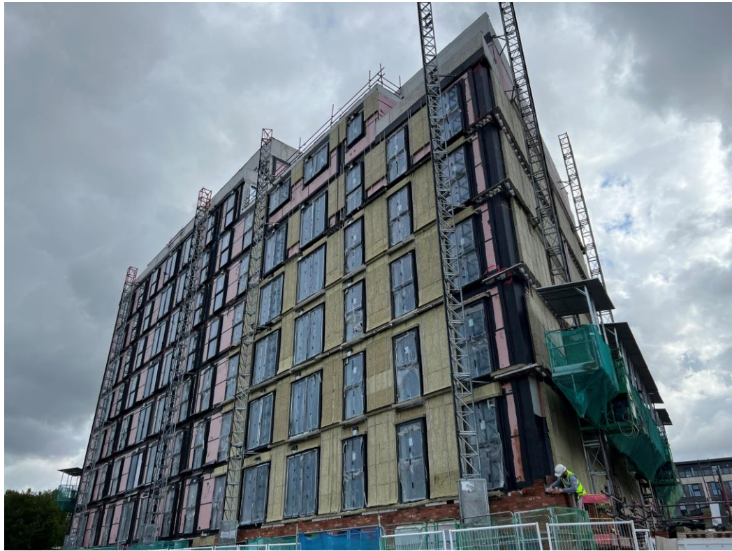
Worrall Street site view
