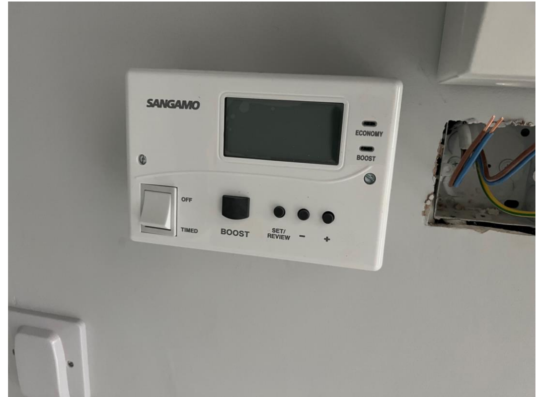
Level 2 – 2 nd fix electrical
