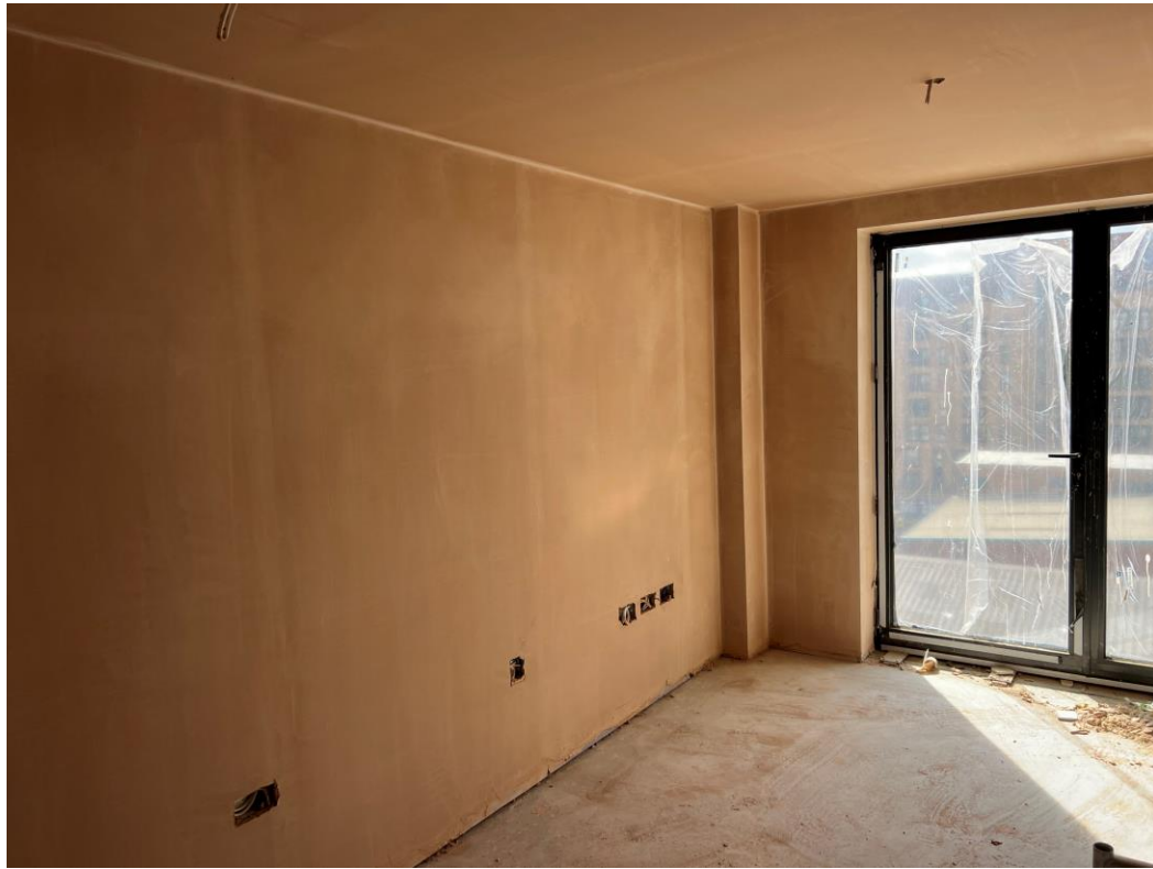
Level 5 - apartments plaster skimmed
