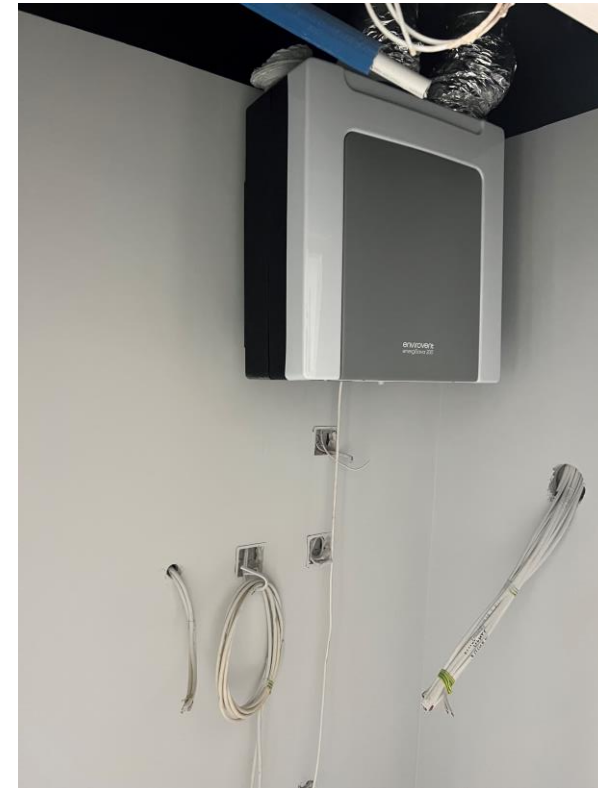
Level 5 – 2 nd fix mechanical installation
