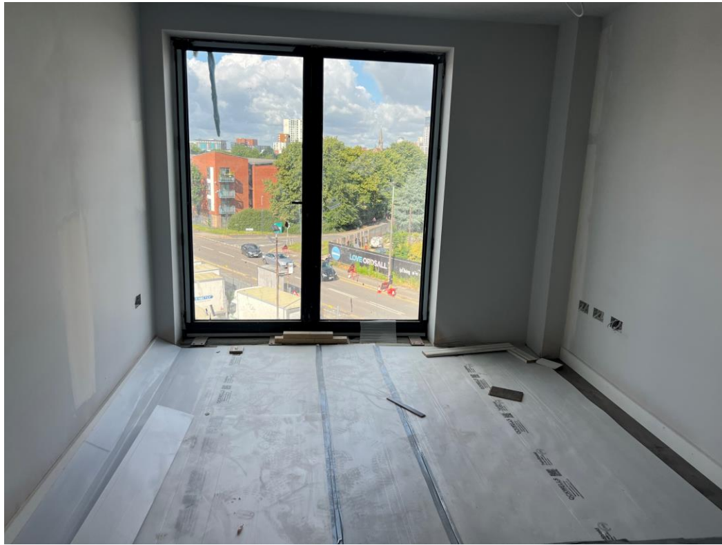
Level 4 – Laminate flooring installed
