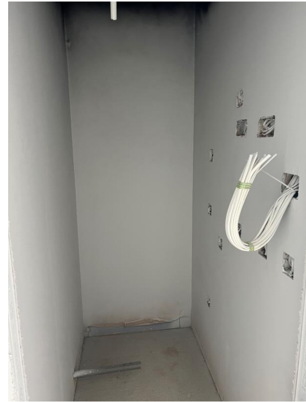
Level 6 – Apartment decoration walls and ceiling
