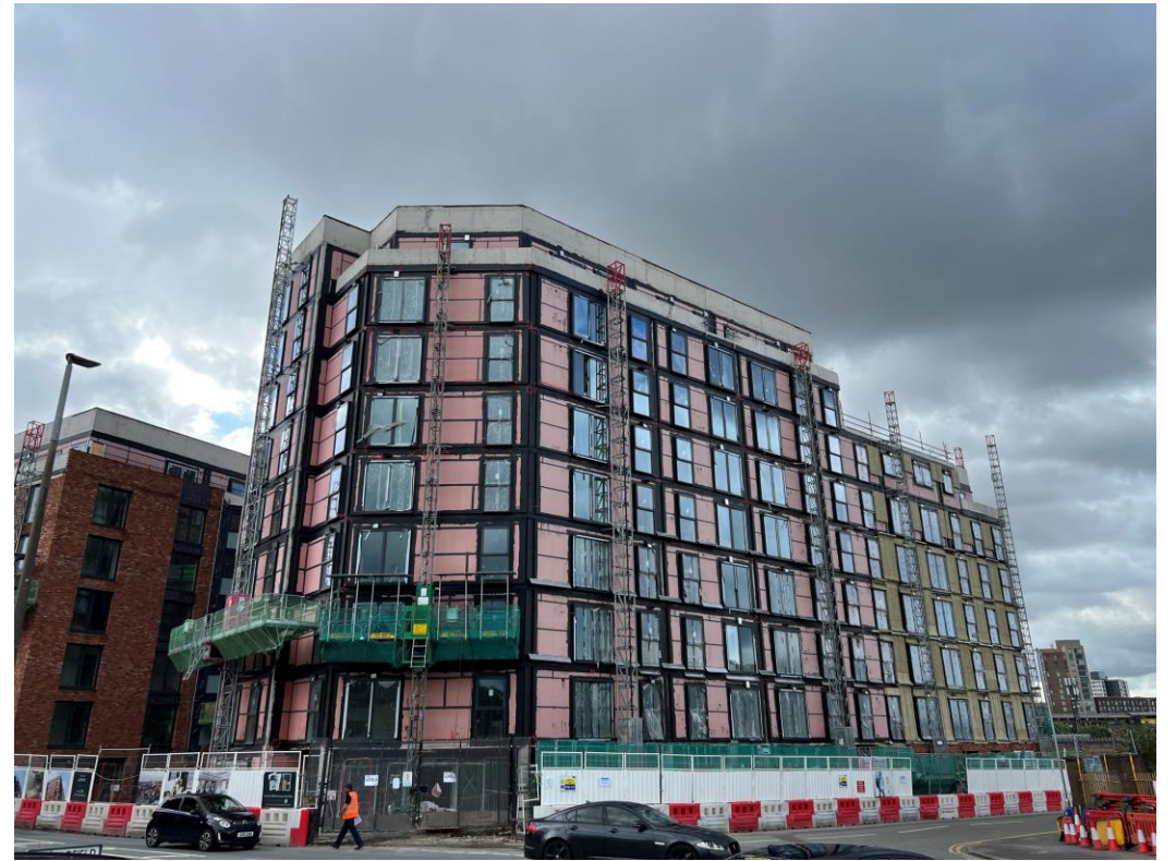
Ordsall Lane site view
