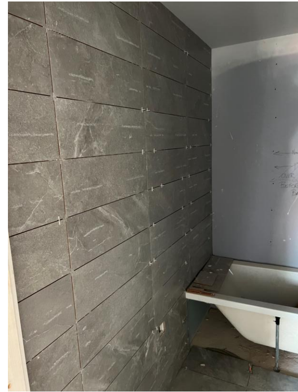
Level 4 – wall and floor tiling
