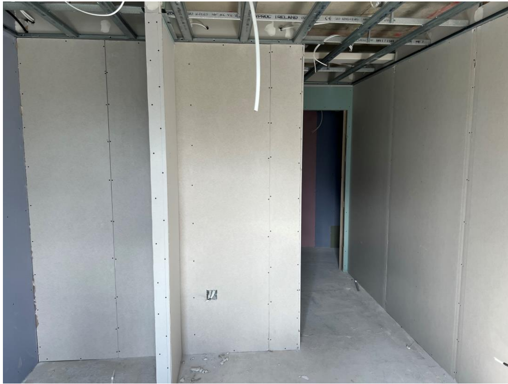
Level 8 – apartment walls and ceilings formed
