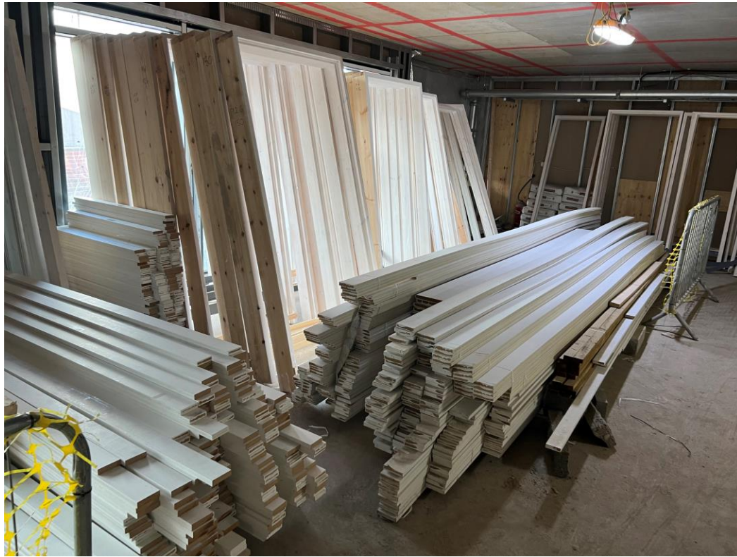
Door frames and skirting storage
