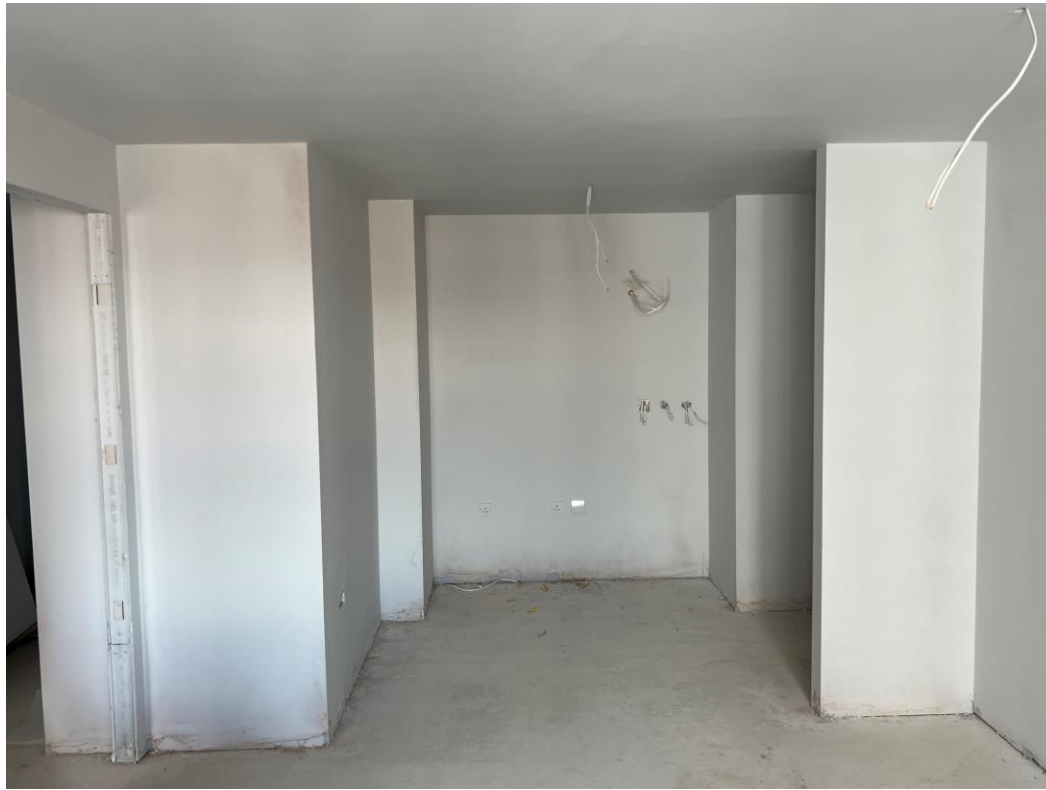
Level 6 – corridor and apartment walls formed
