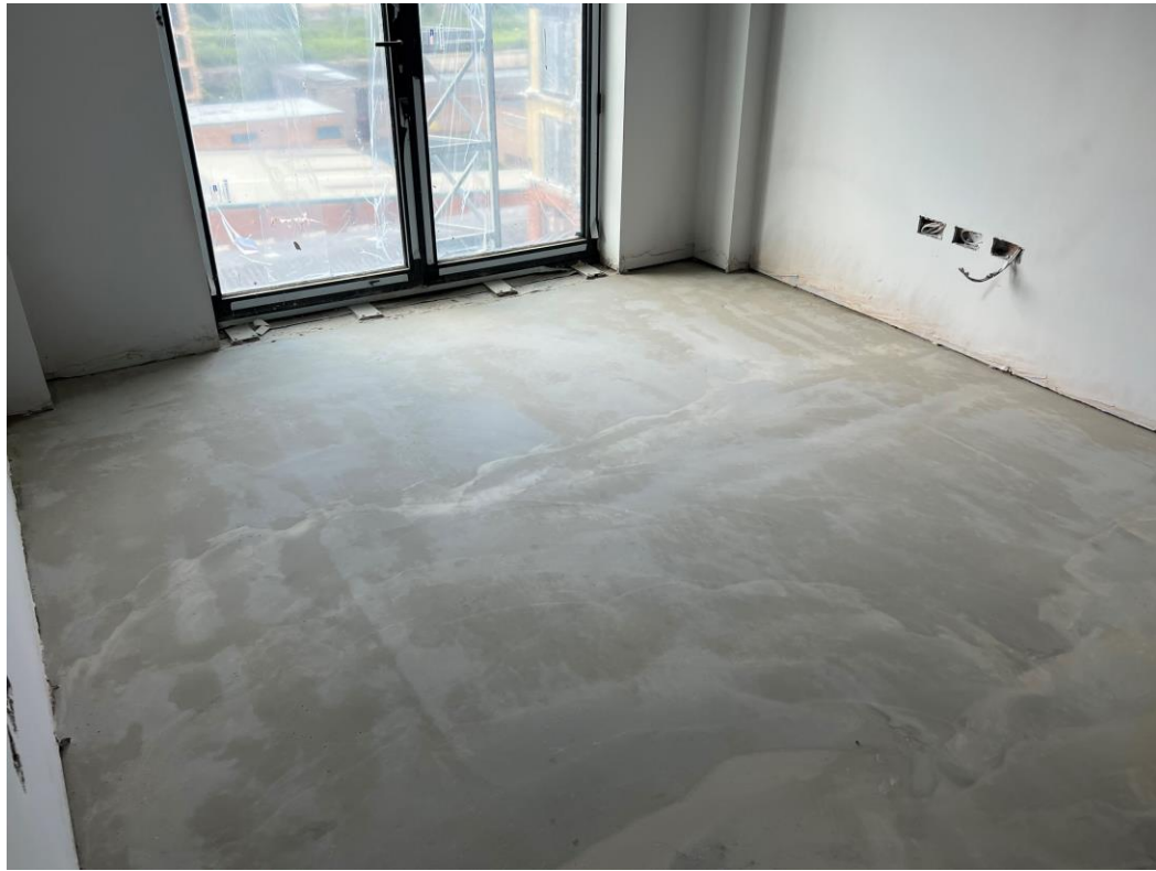
Level 6 – latex screed floors
