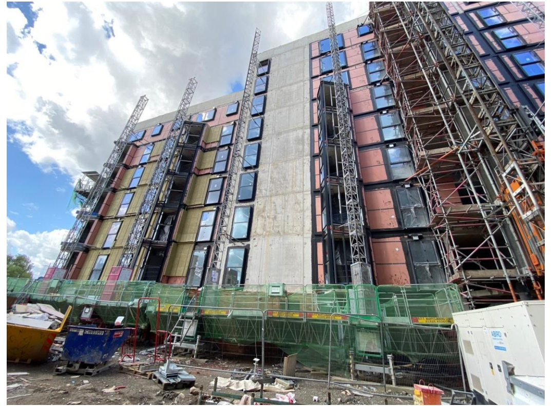
Block A wall insulation and brickwork
