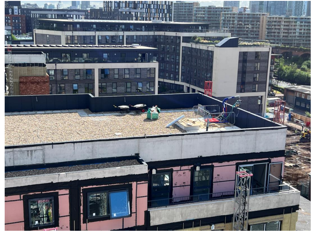
Block B inverted main roof system complete
