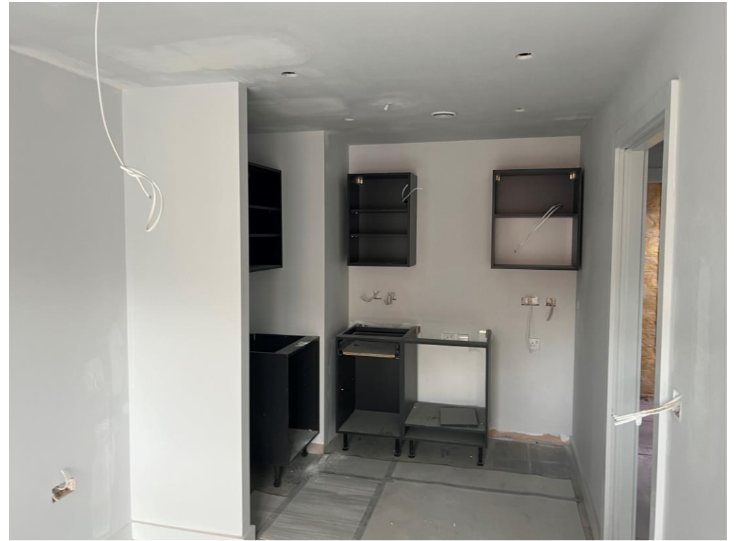
Level 1 – Kitchen units installed
