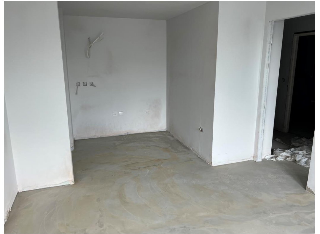
Level 6 – latex screed floors
