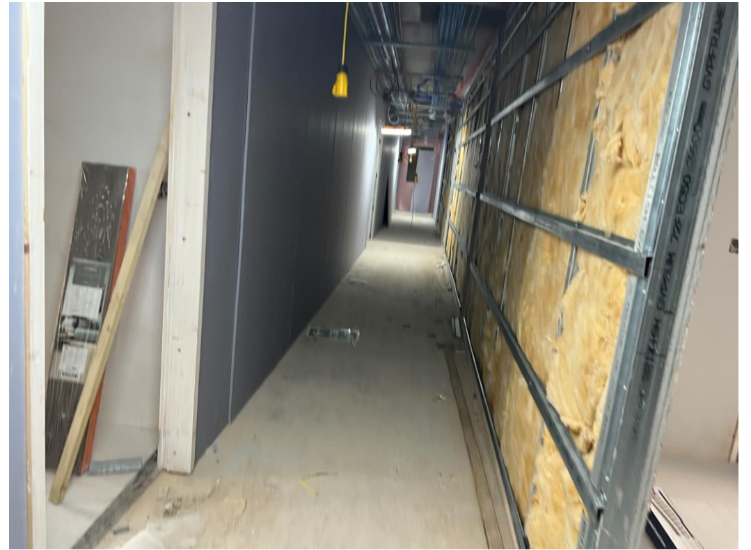
Level 6 – corridor and apartment walls formed
