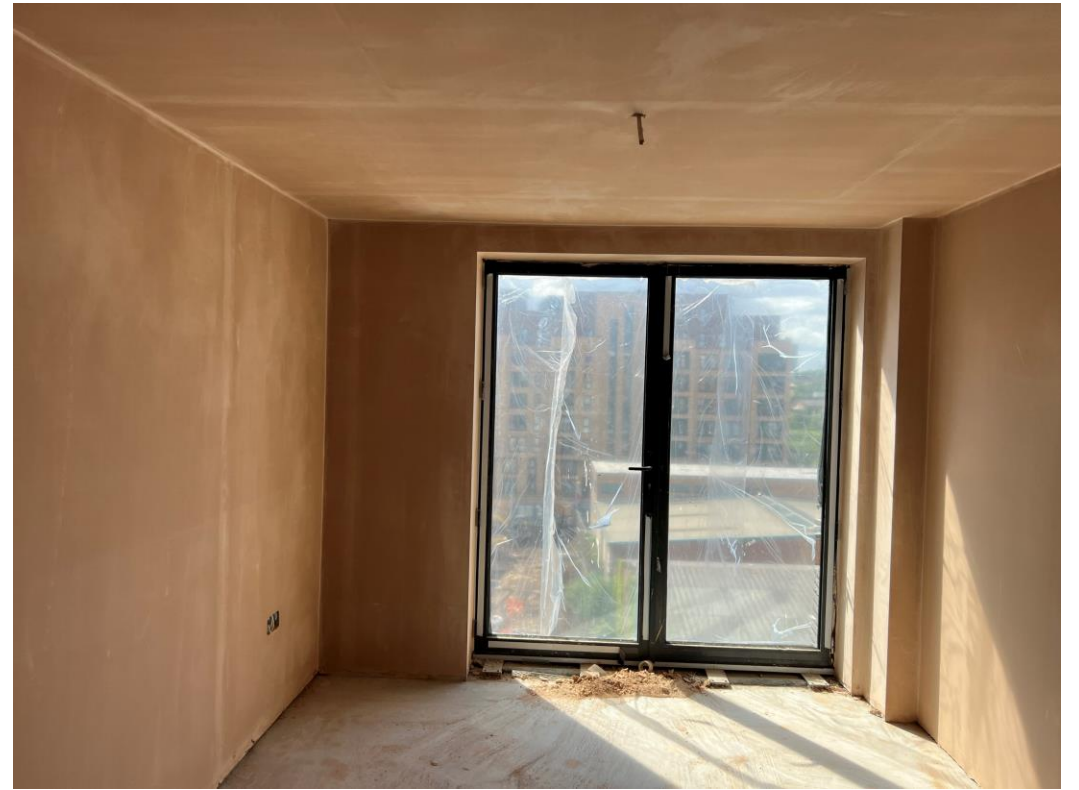
Level 5 - apartments plaster skimmed
