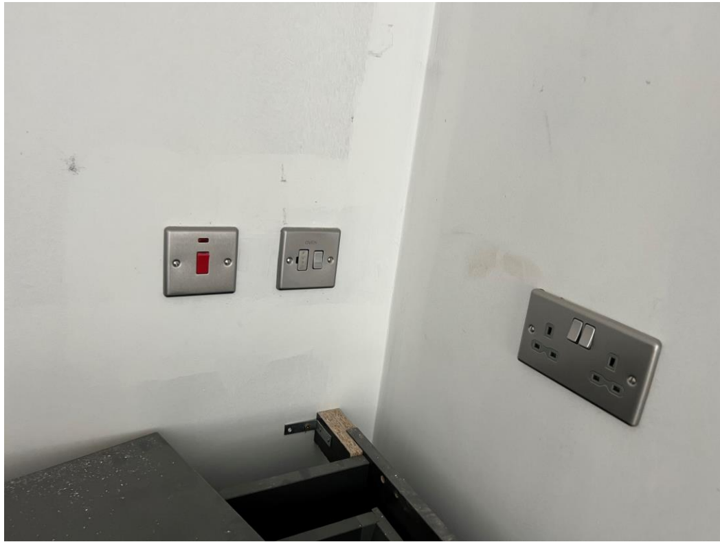
Level 2 – 2 nd fix electrical sockets
