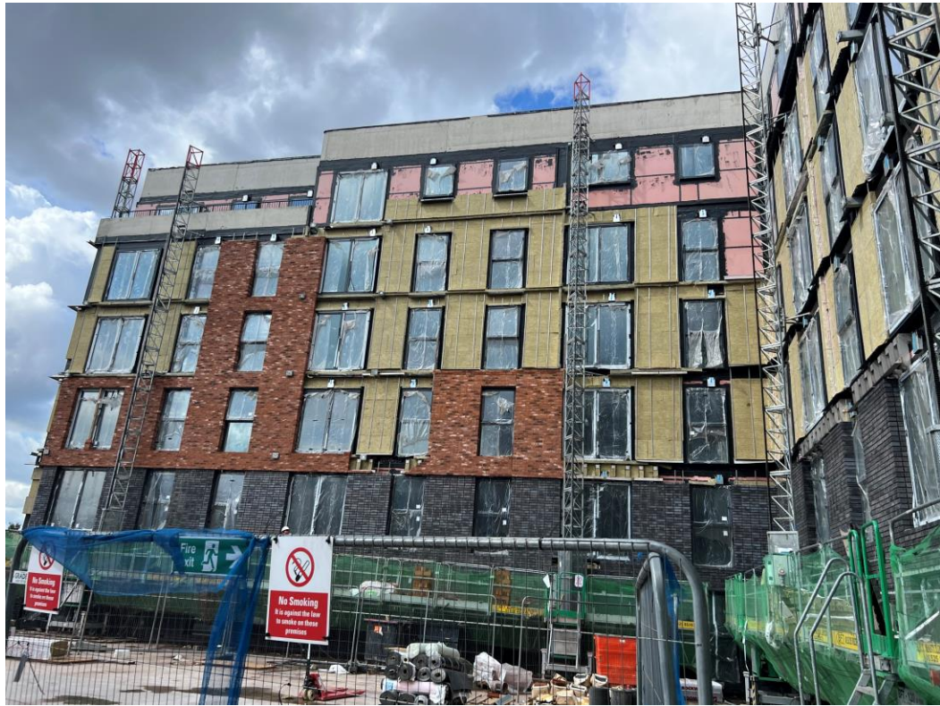
Block B wall insulation and brickwork
