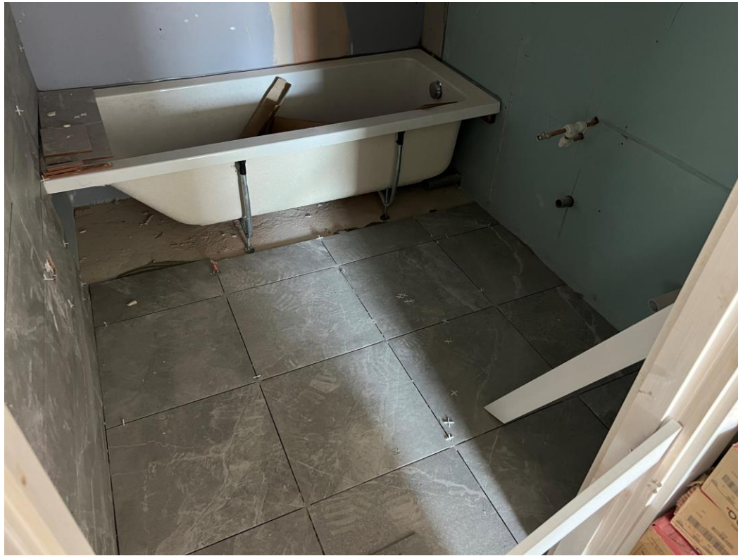
Level 4 – wall and floor tiling
