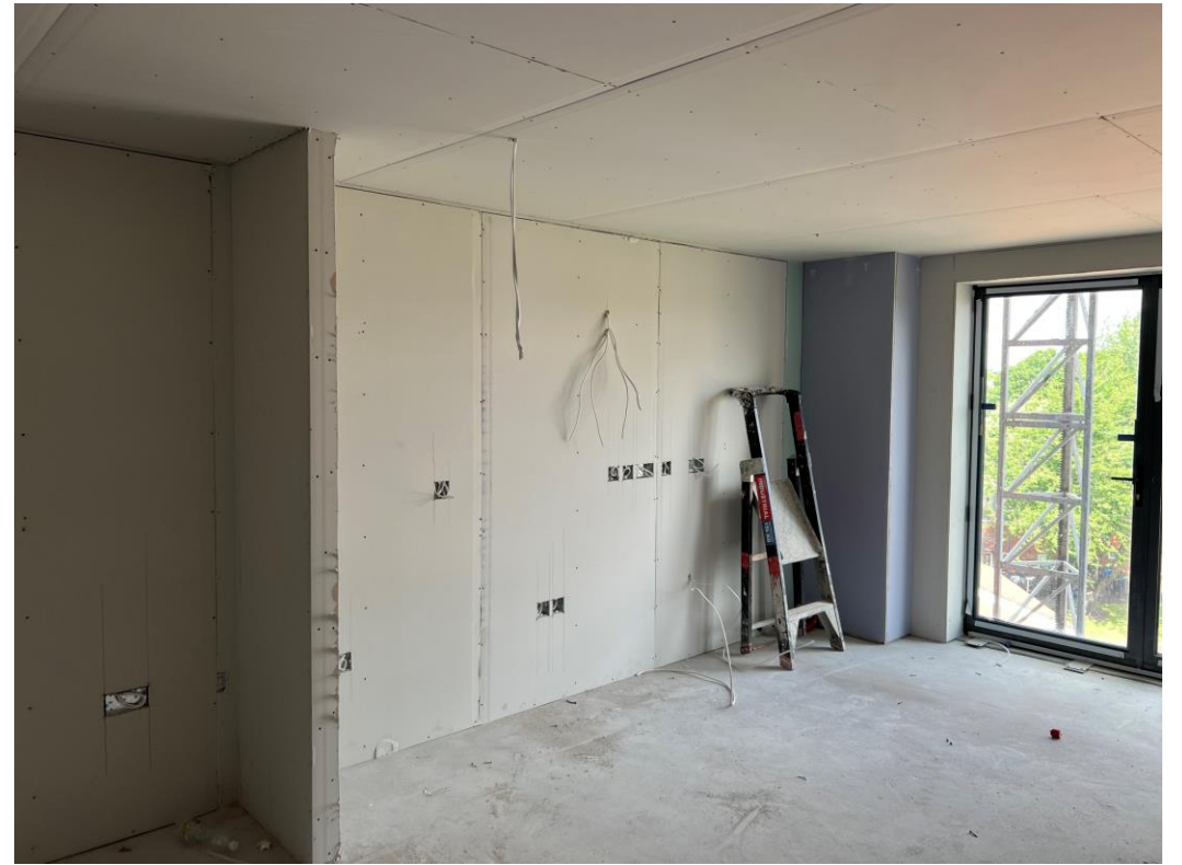
Level 5 – apartments prepared for plastering
