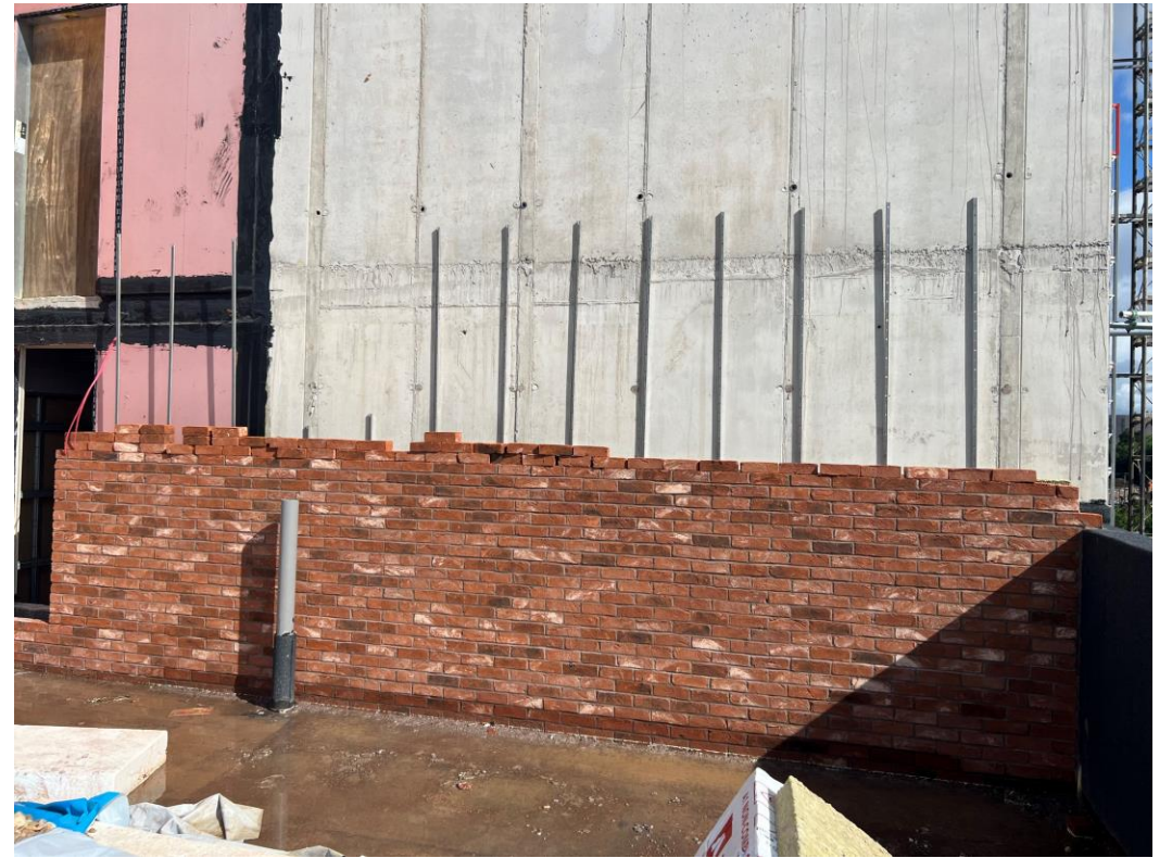
Block A wall insulation and brickwork
