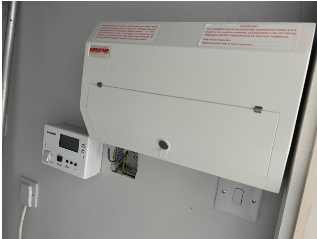
Level 2 – 2 nd fix electrical
