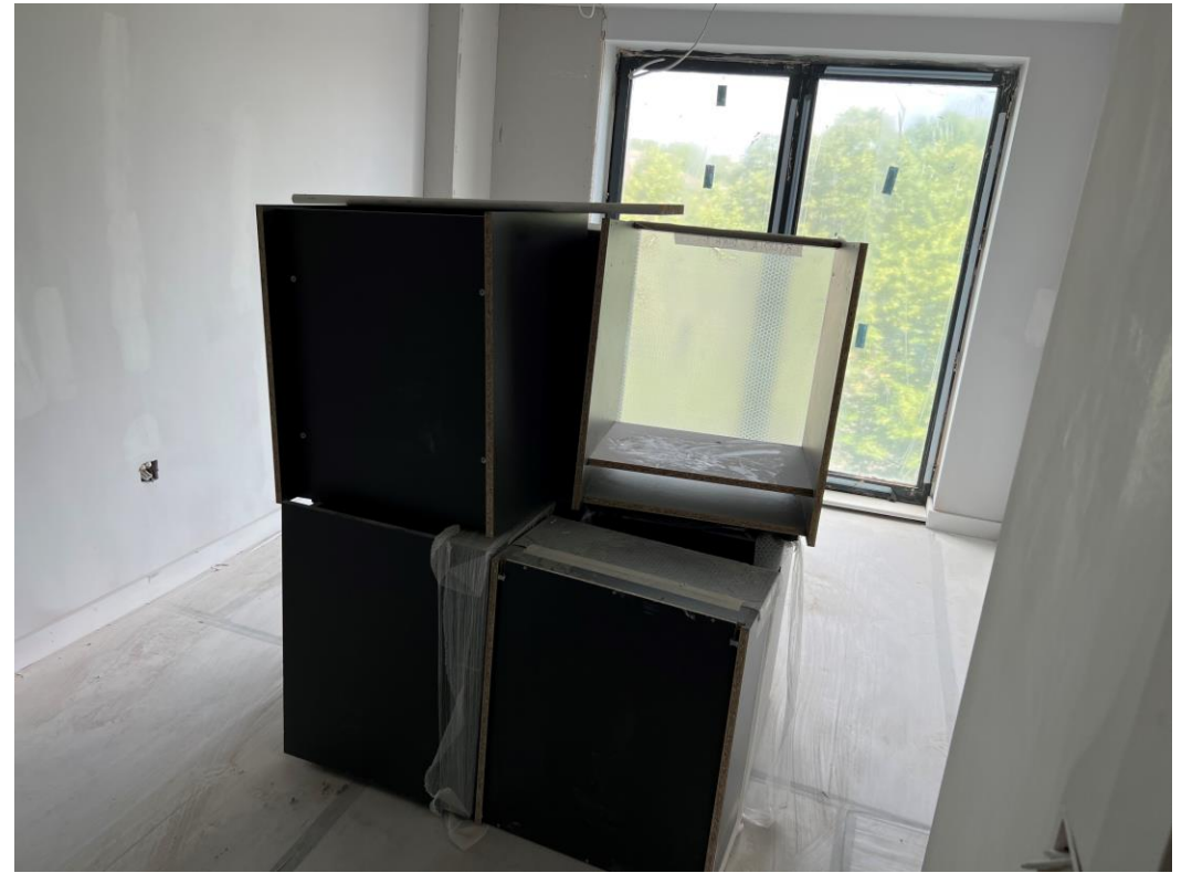
Level 3 – Kitchen units loaded for installation
