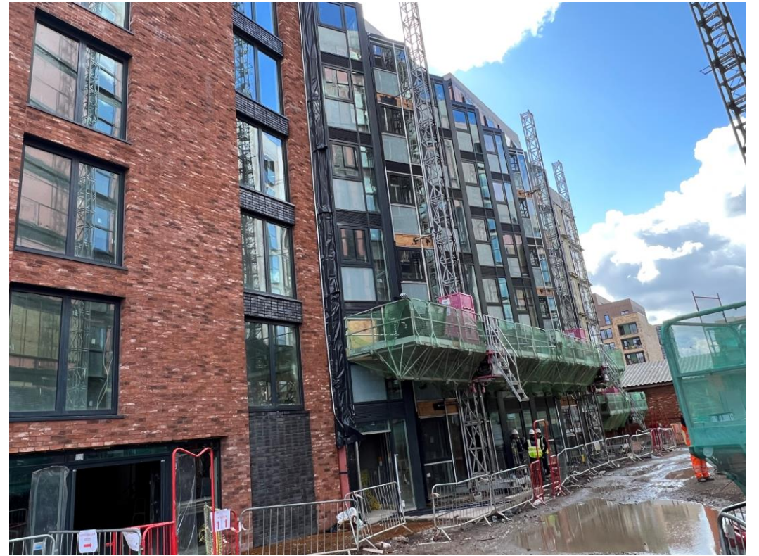
Block B Curtain walling and brickwork
