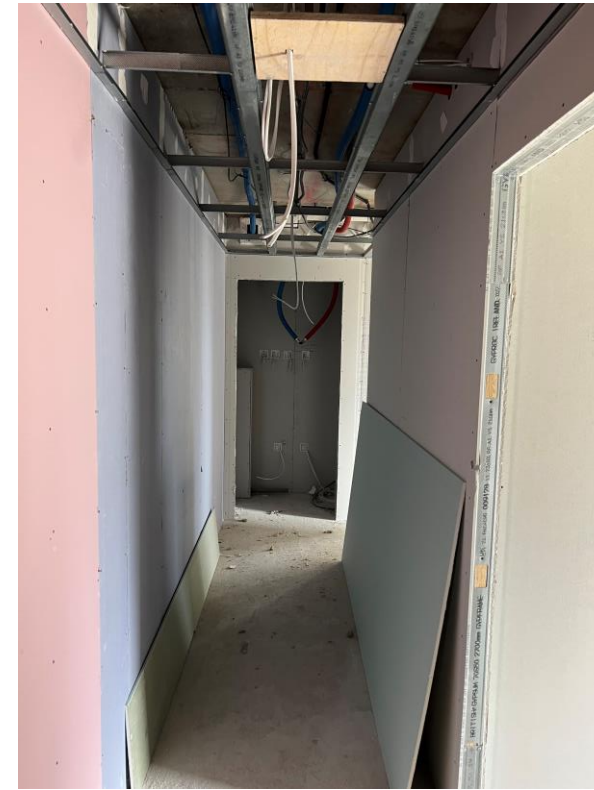
Level 8 – apartment walls and ceilings formed
