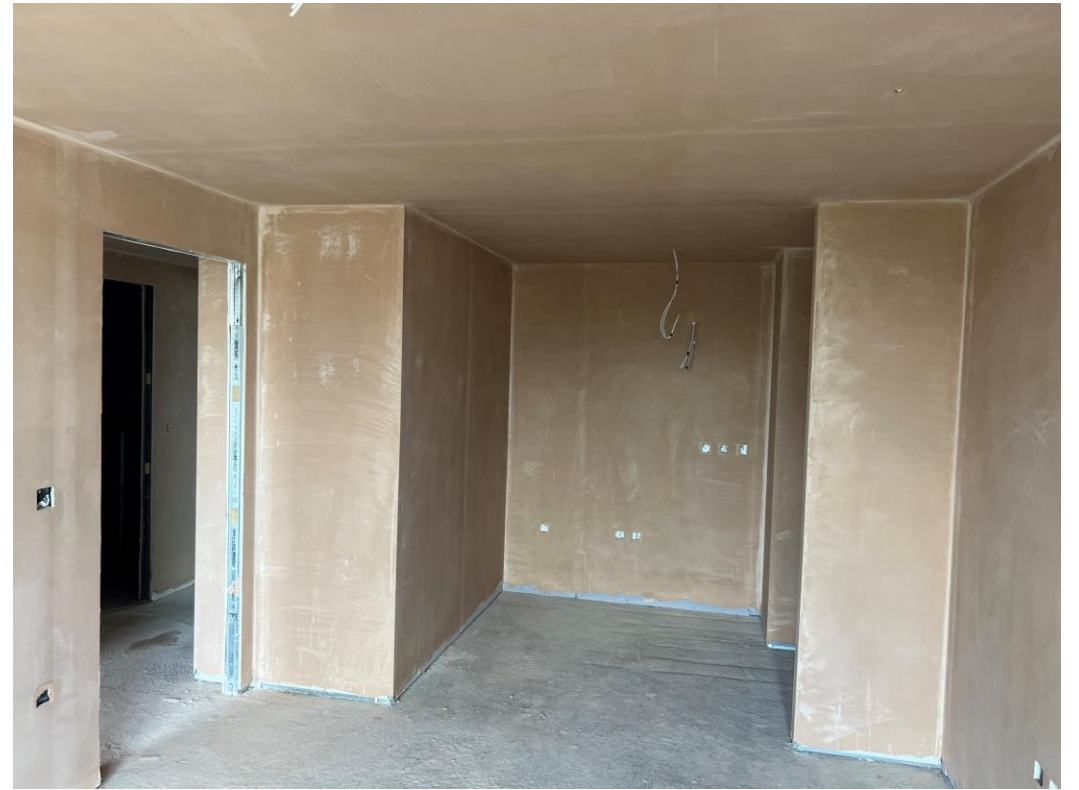
Level 7 – walls and ceilings plastered
