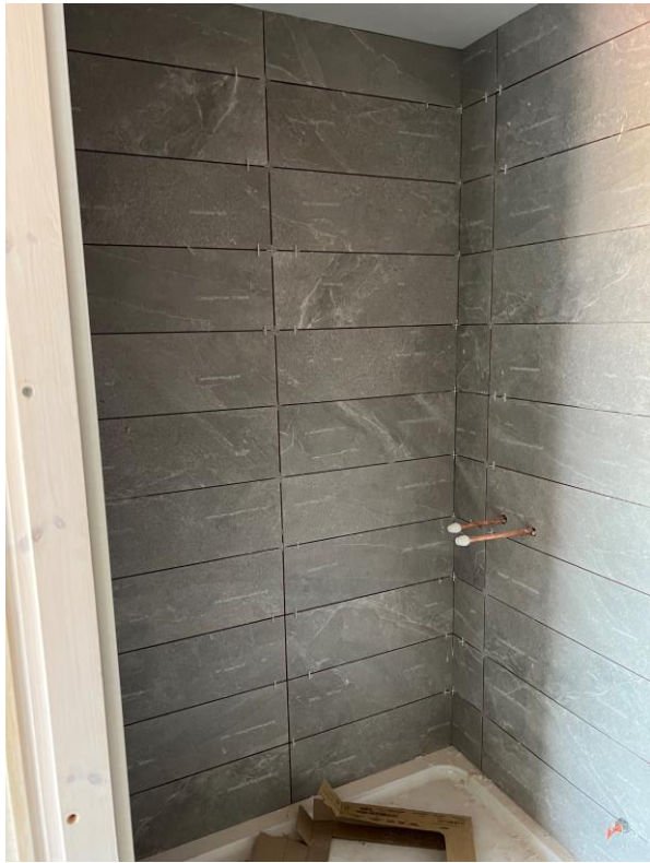
Level 4 – wall and floor tiling
