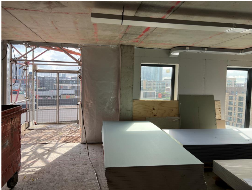
Level 8 – hoist access
