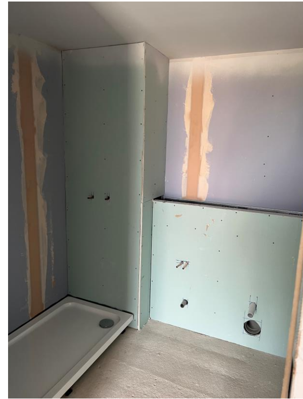
Level 6 – IPS formed & sanitary installation
