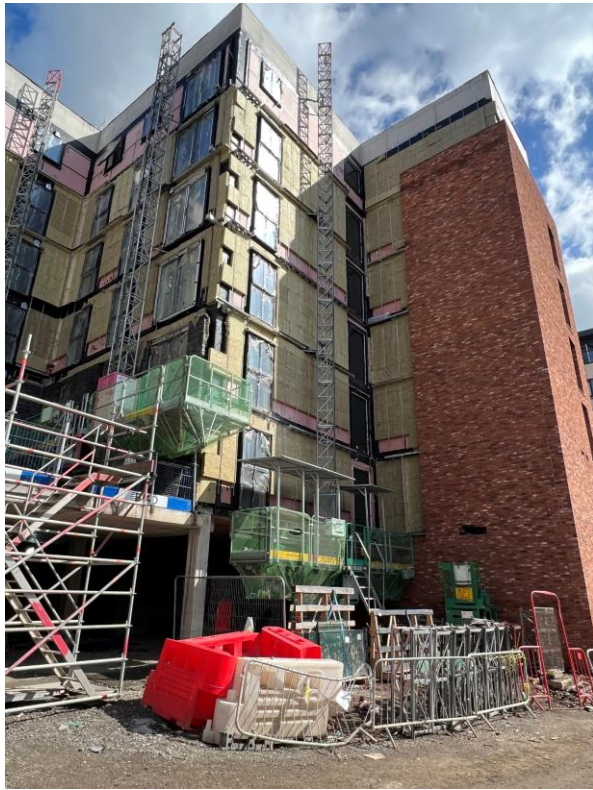
Block B wall insulation and brickwork
