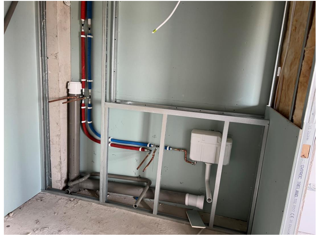
Level 8 – first fix plumbing
