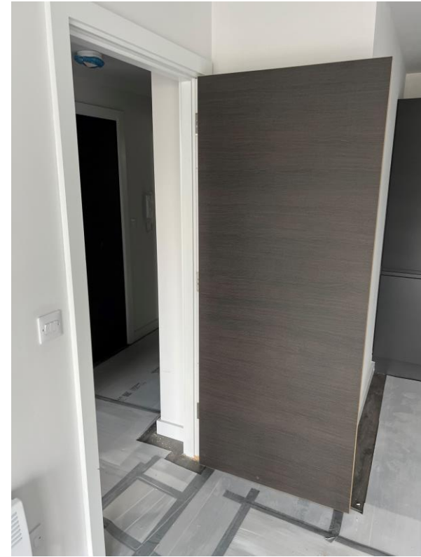
Level 1 – doors installed
