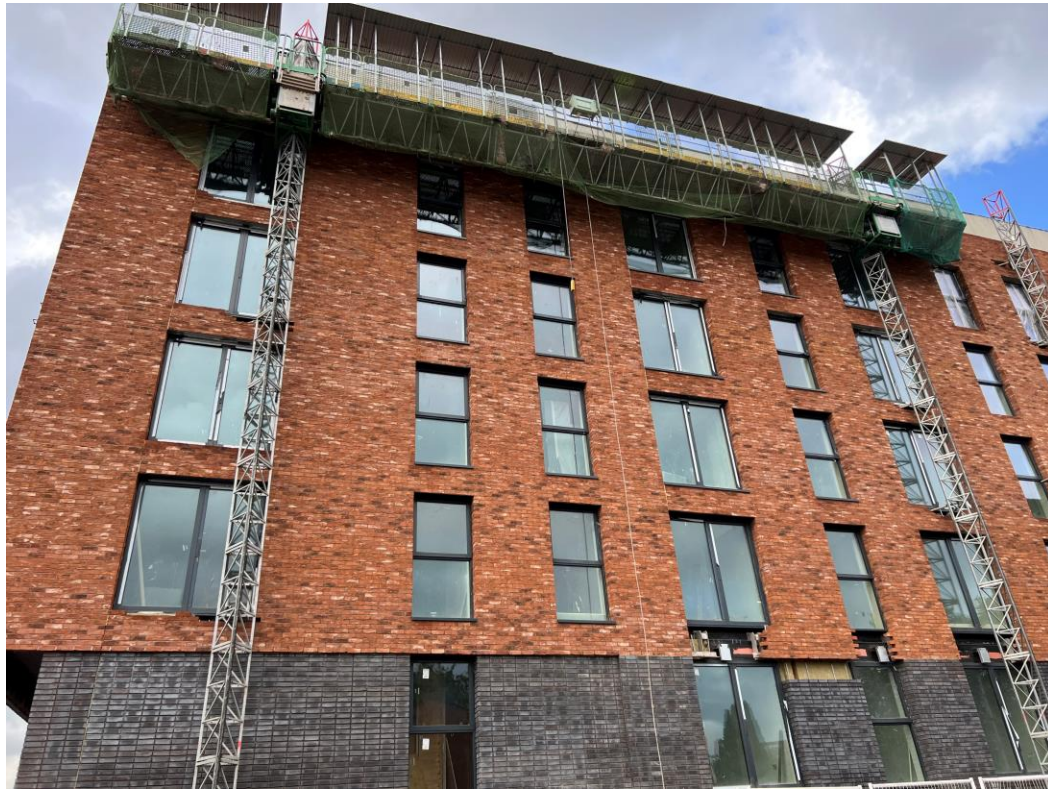
Ordsall Lane site view
