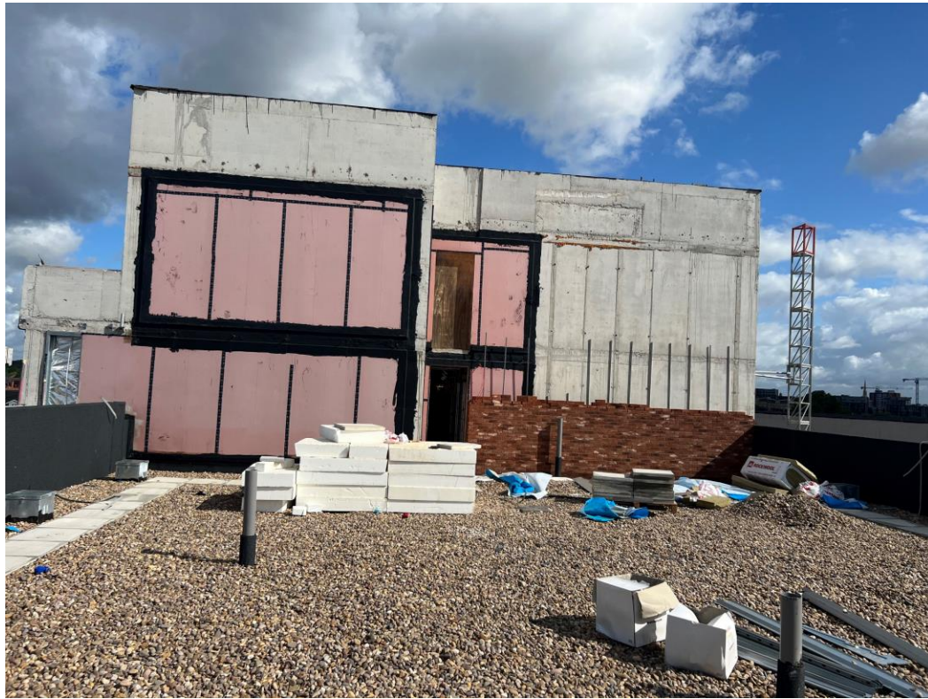
Block A wall insulation and brickwork
