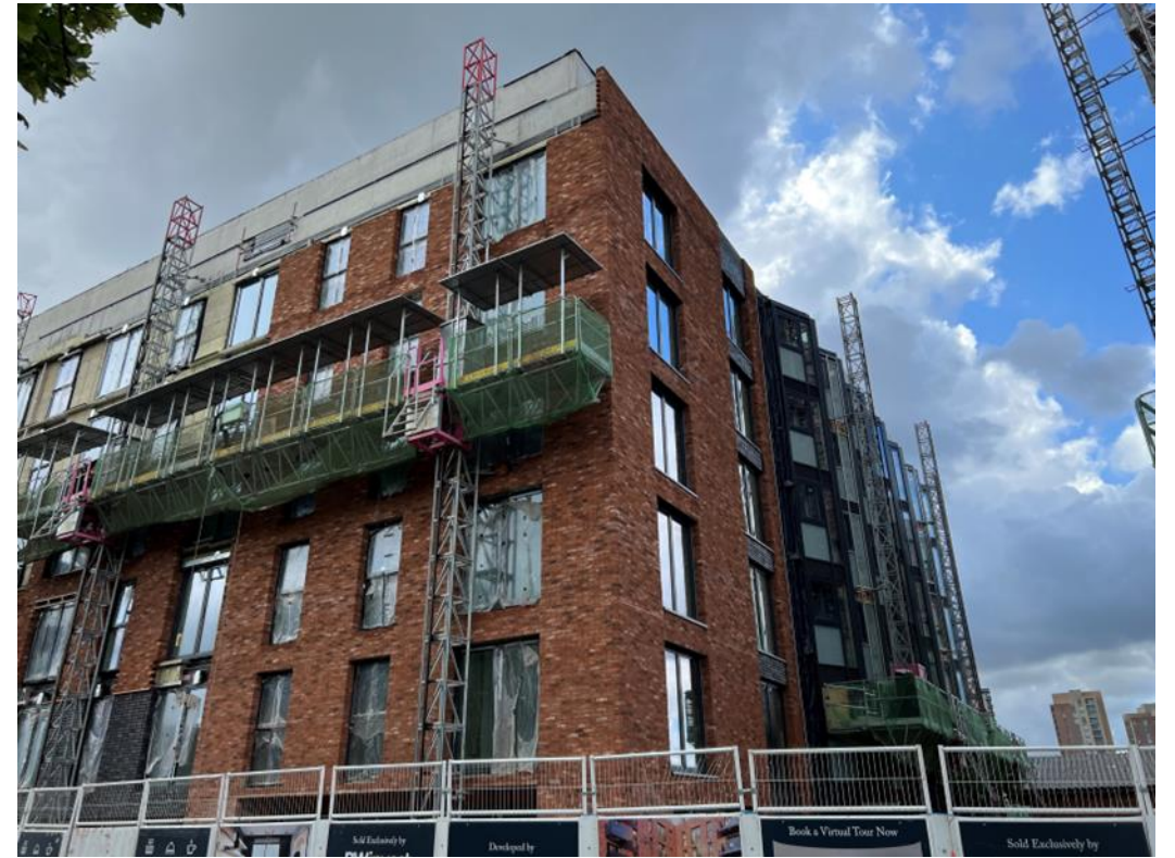
Ordsall Lane site view
