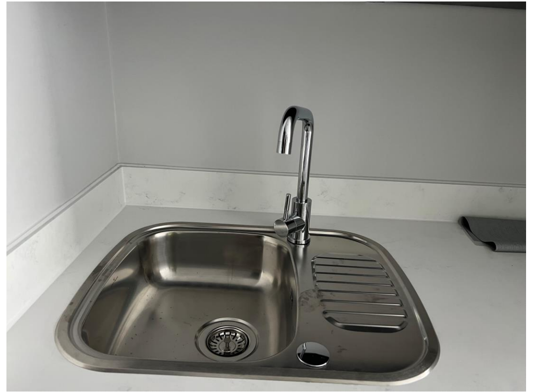
Level 1 – kitchen complete
