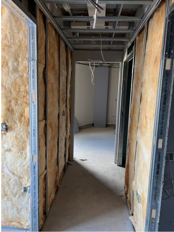
Level 8 – corridor and apartment walls formed
