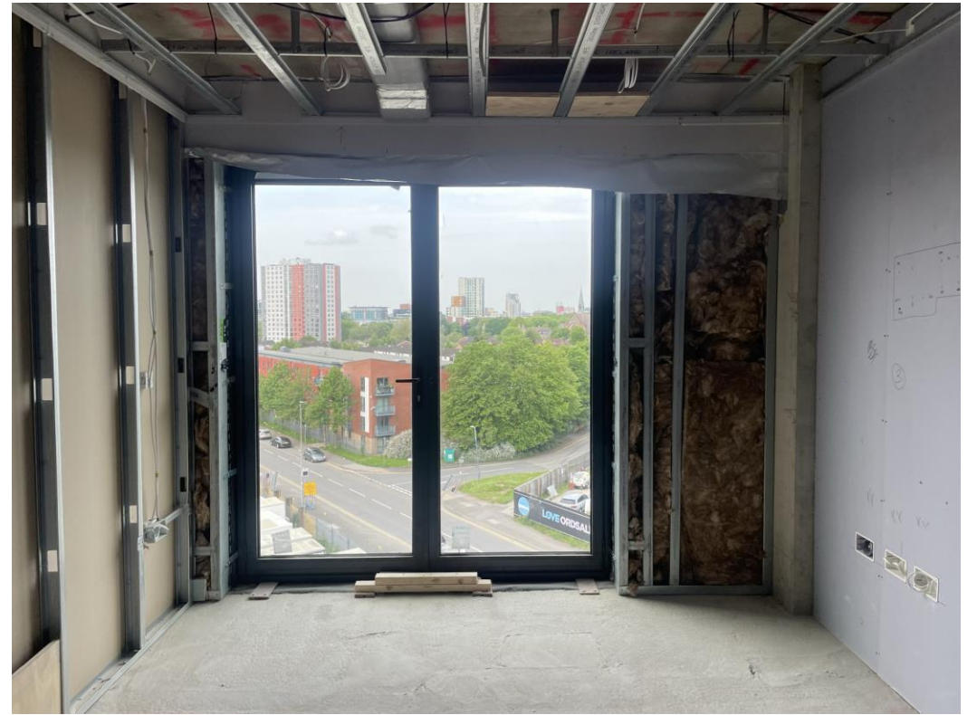
Level 6 – corridor and apartment walls formed
