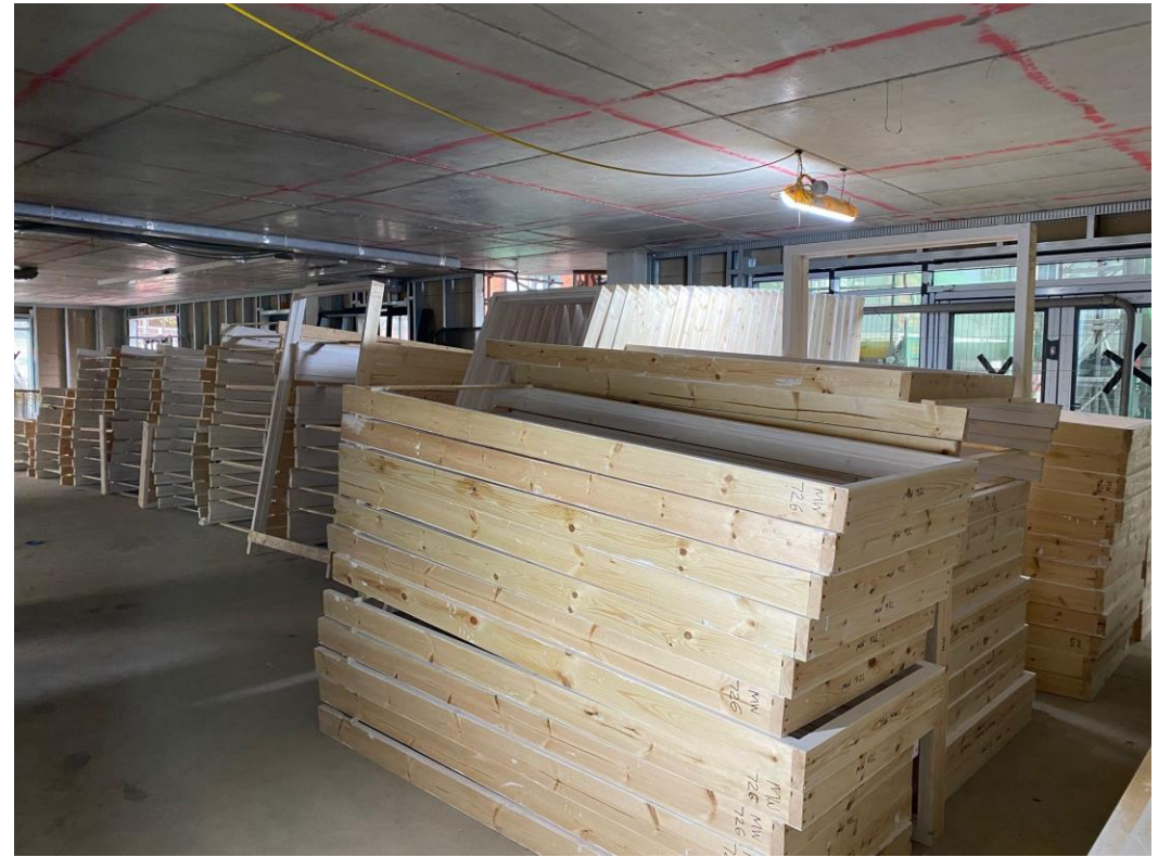
Apartment doorframes stored
