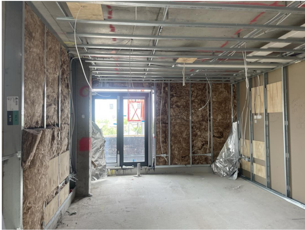
Level 6 – corridor and apartment walls formed
