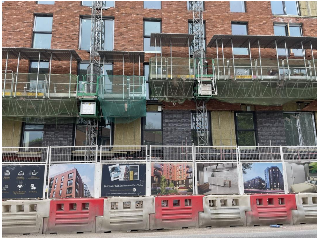
Ordsall Lane site view
