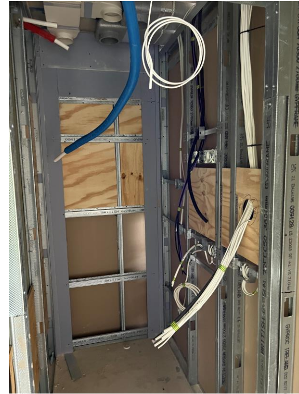
Level 5 – 1 st fix electrical
