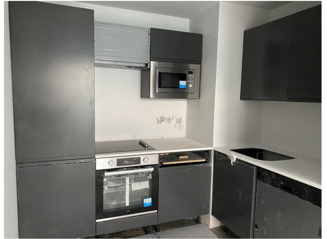
Level 1 – Kitchen installed
