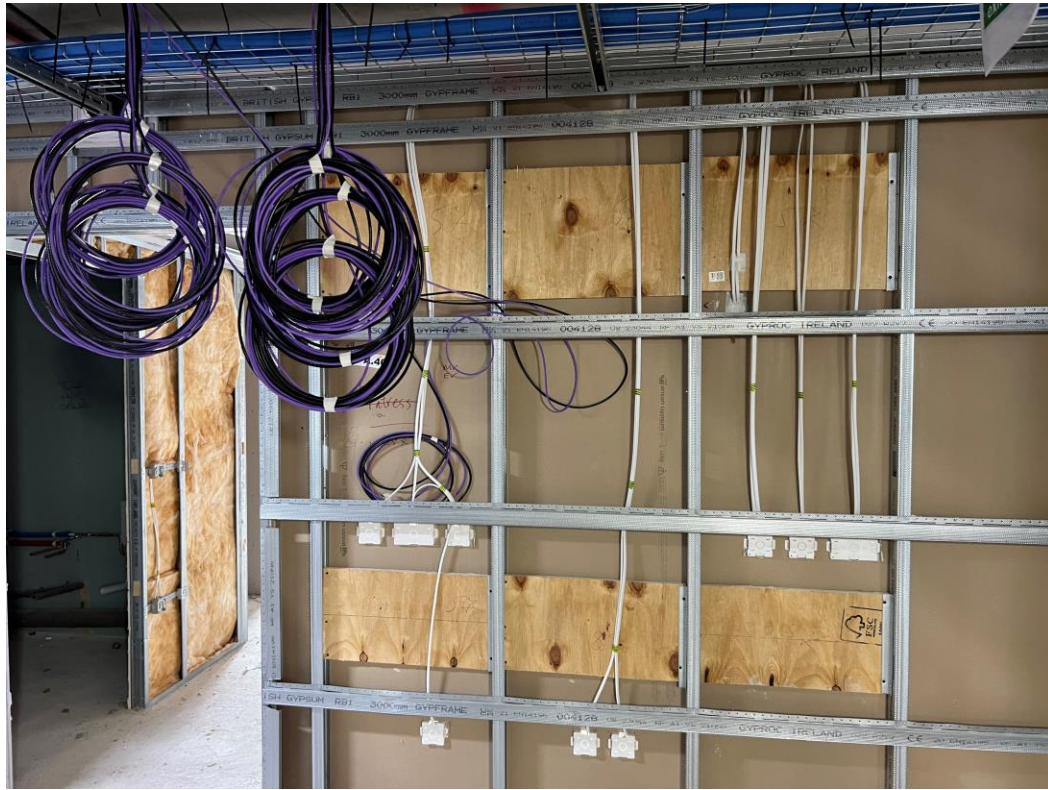
Level 4 – 1 st fix electrical
