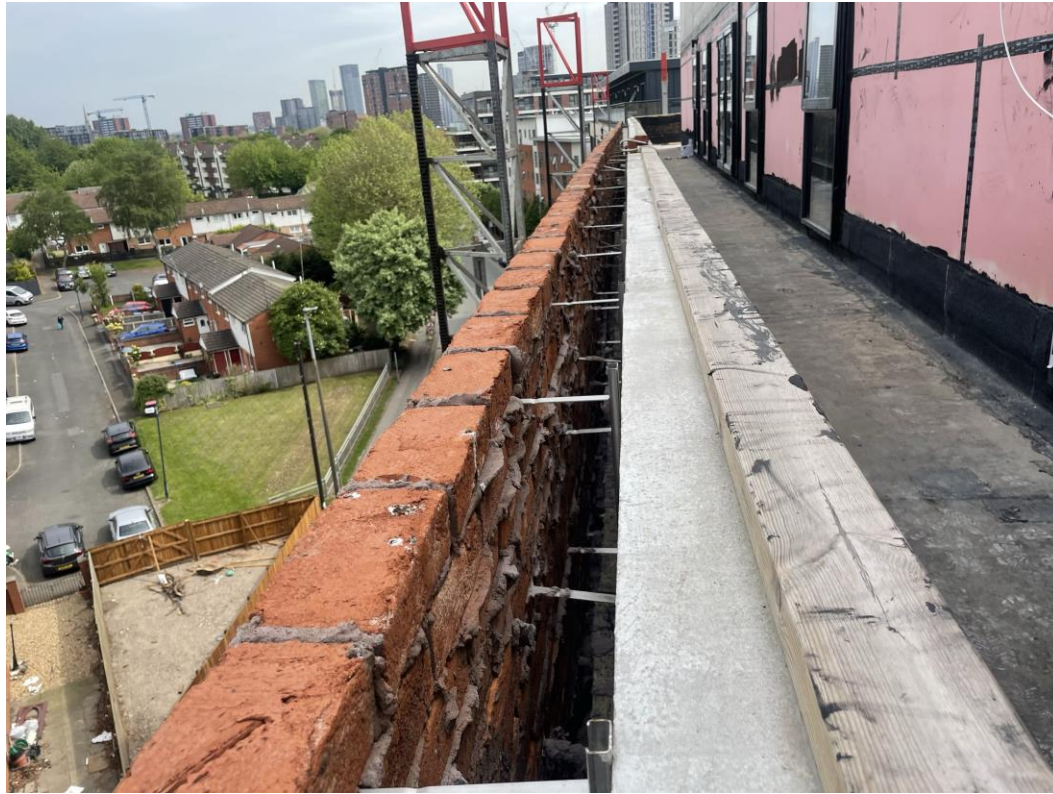
Block B parapet brickwork
