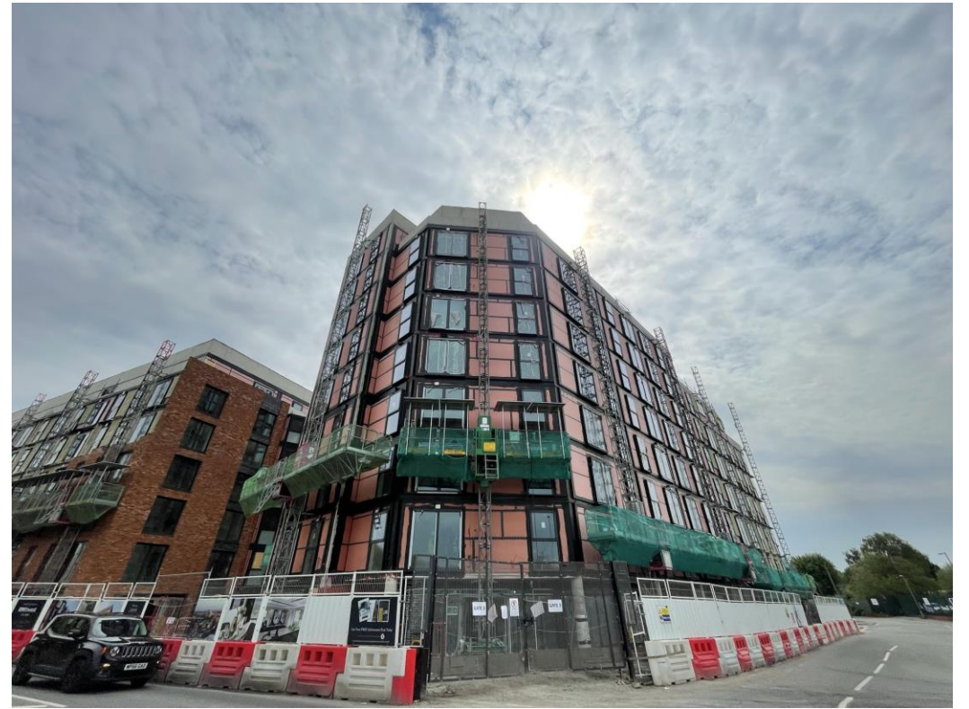
Ordsall Lane site view
