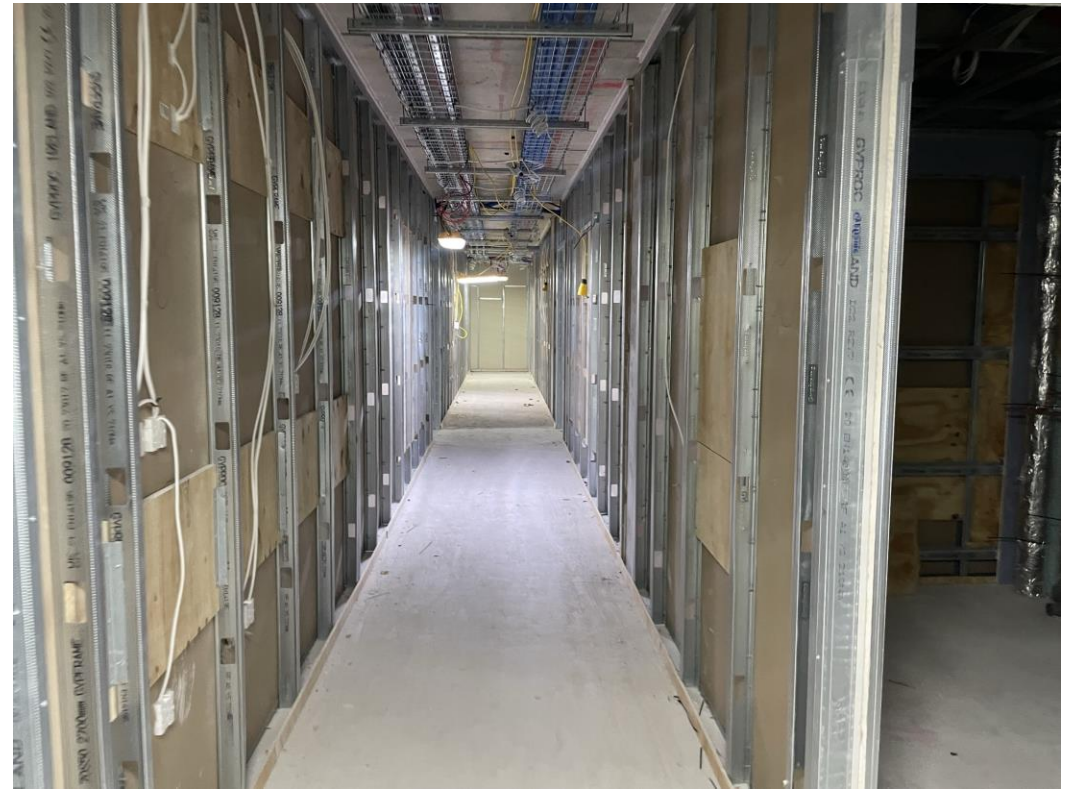
Level 5 – corridor and apartment walls formed
