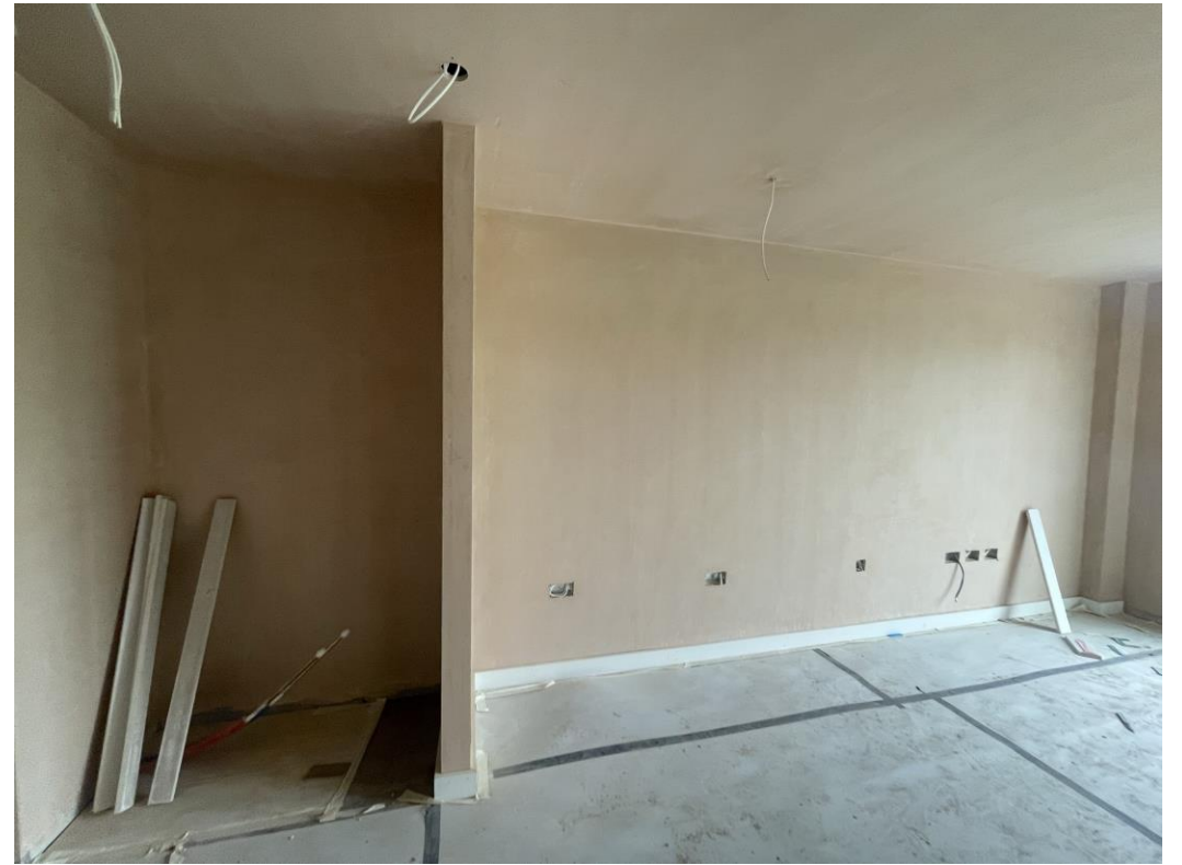
Level 4 - apartments plastered
