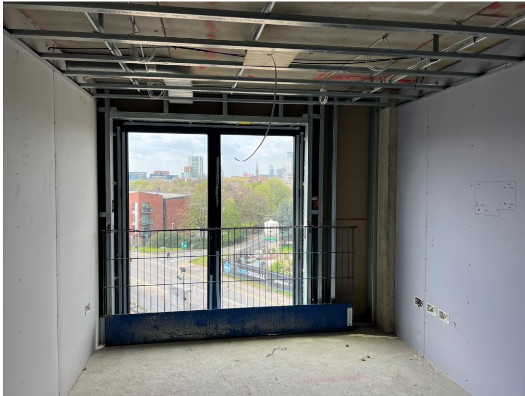
Level 5 – ceiling installation
