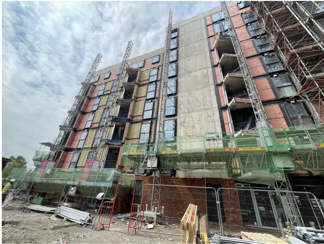
Block A weatherboarding & windows installed
