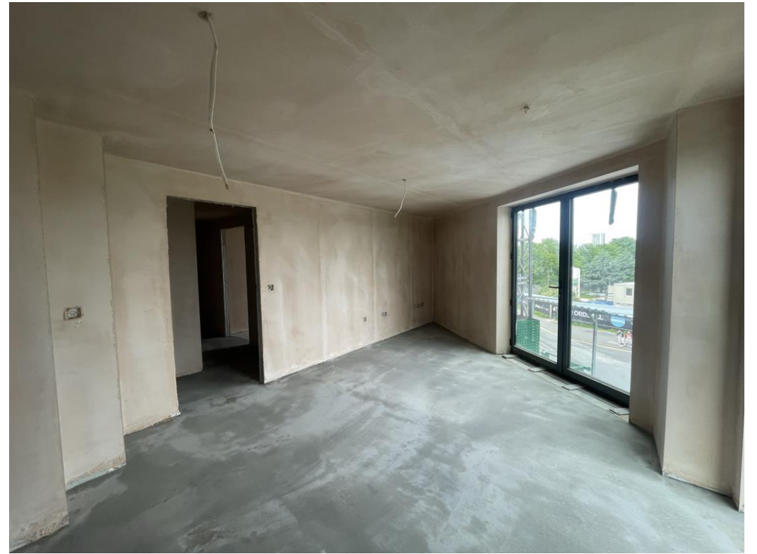
Level 3 – Apartments ready for decoration
