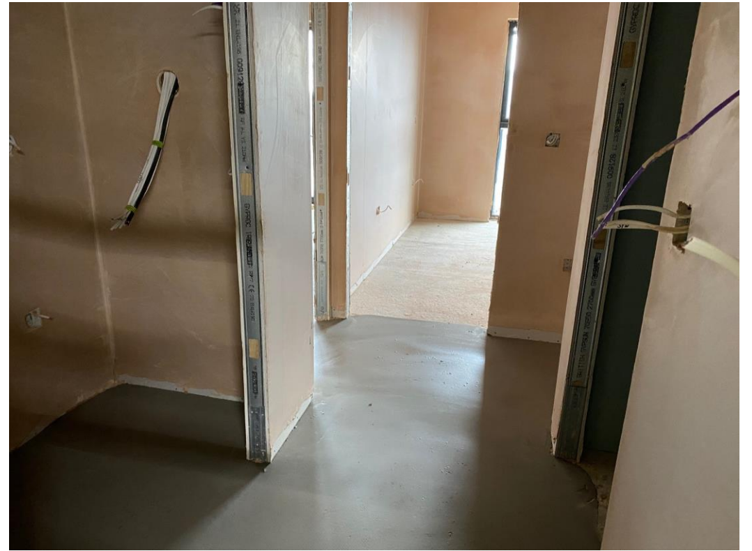
Level 3 – Apartments ready for decoration
