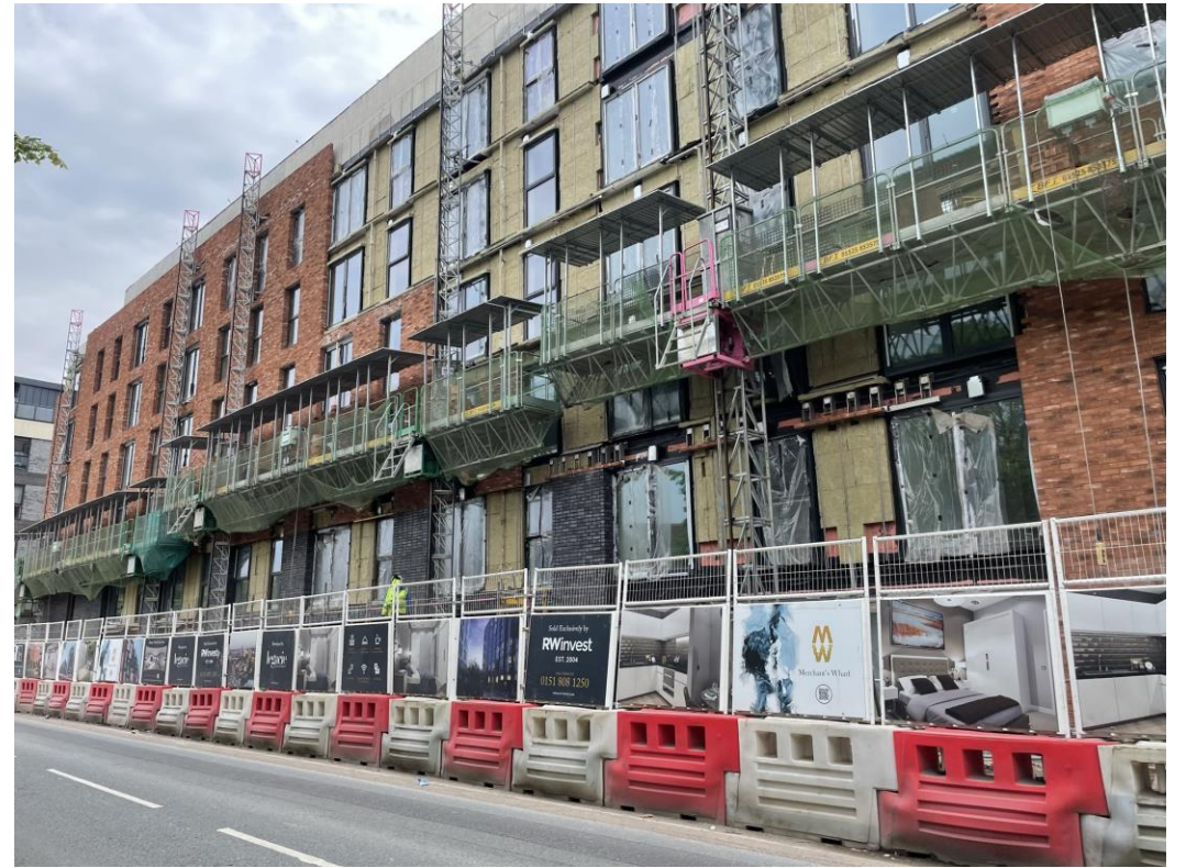
Ordsall Lane site view
