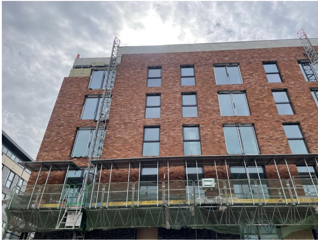
Ordsall Lane site view
