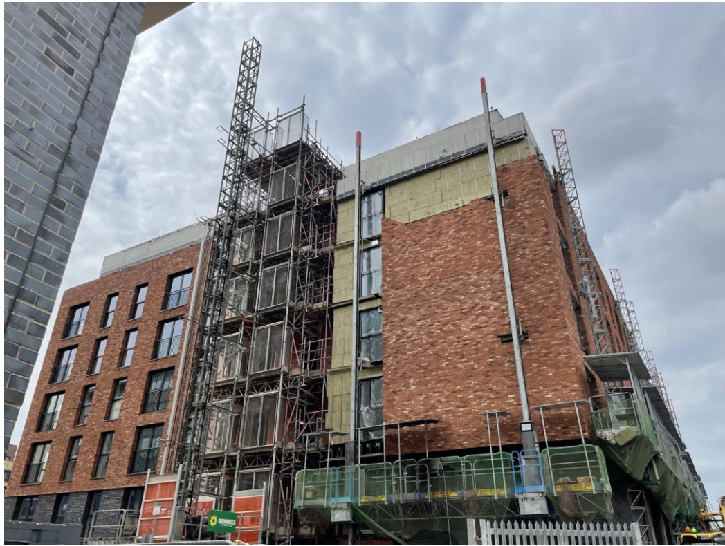
Ordsall Lane site view
