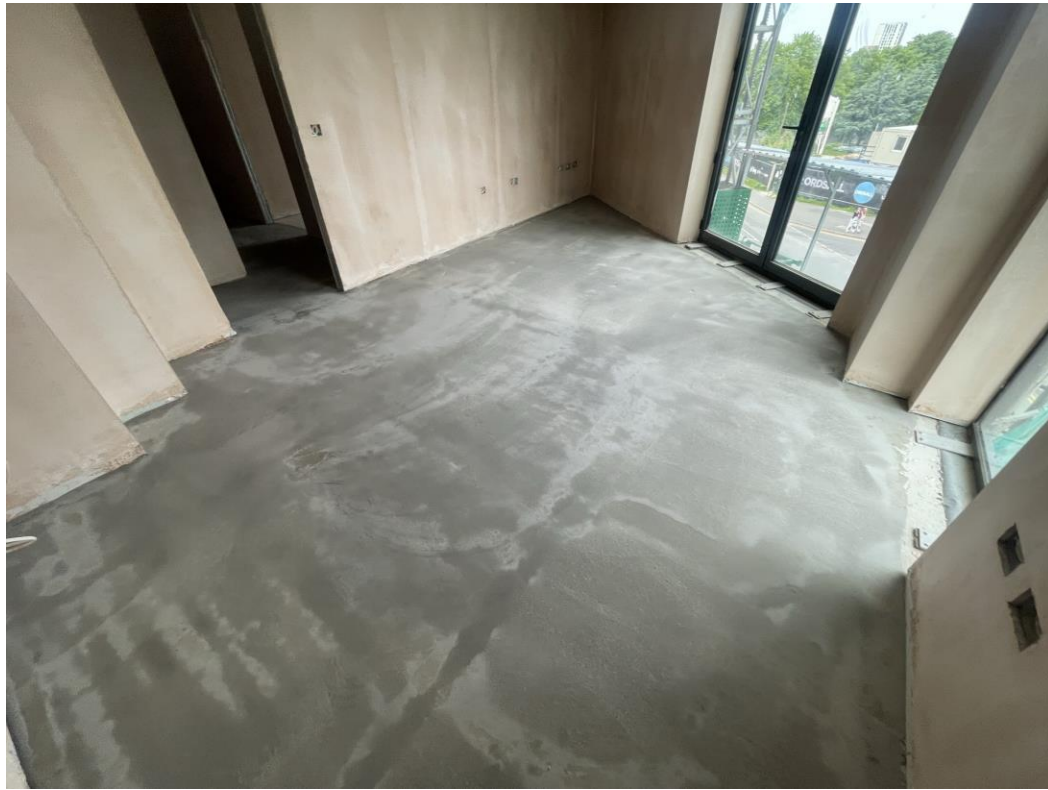
Level 3 – Apartments ready for decoration
