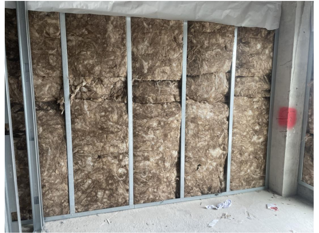
Level 8 – corridor and apartment walls formed
