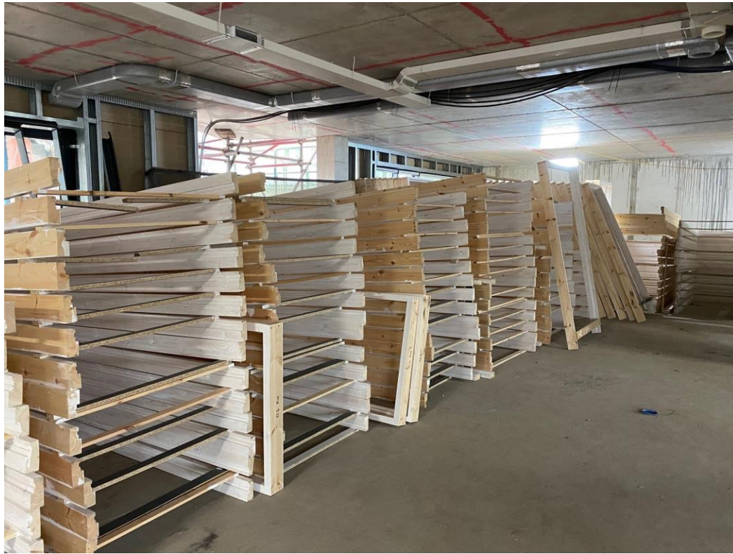
Apartment doorframes stored
