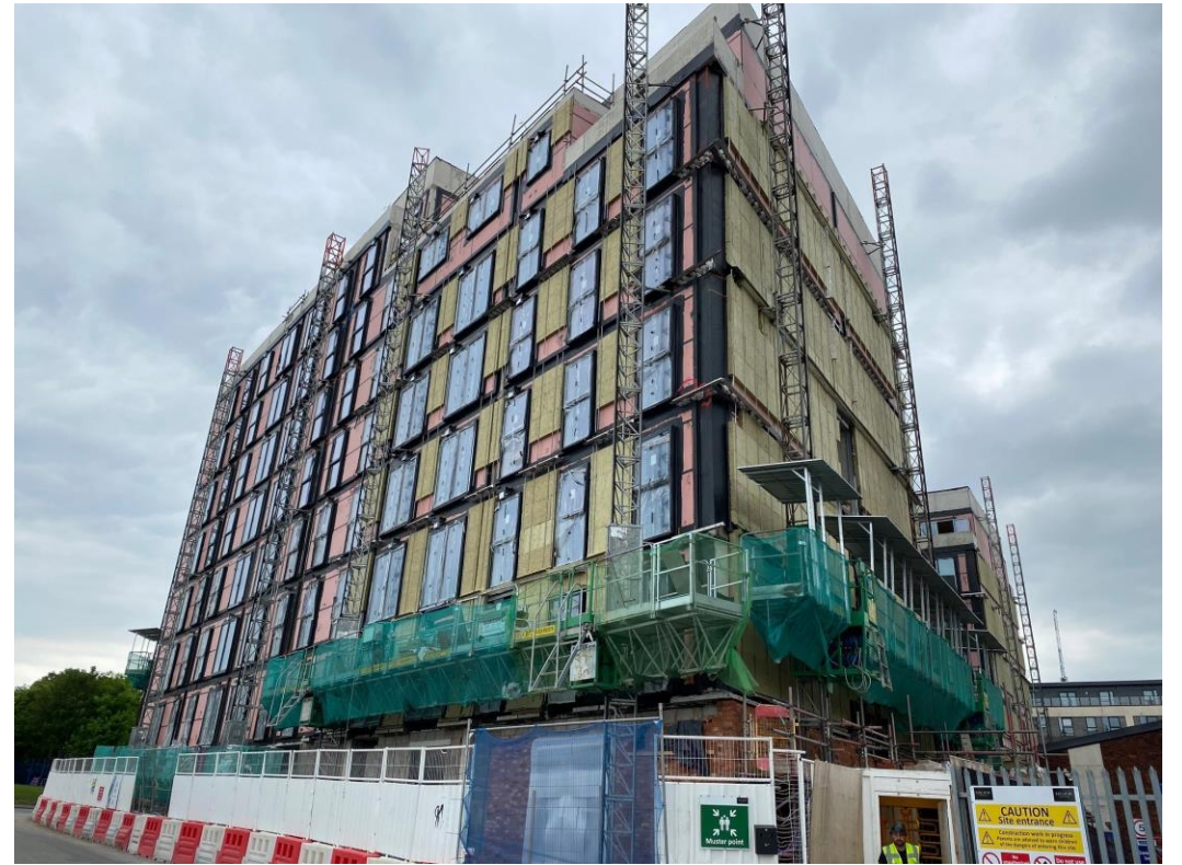
Worrall Street site view
