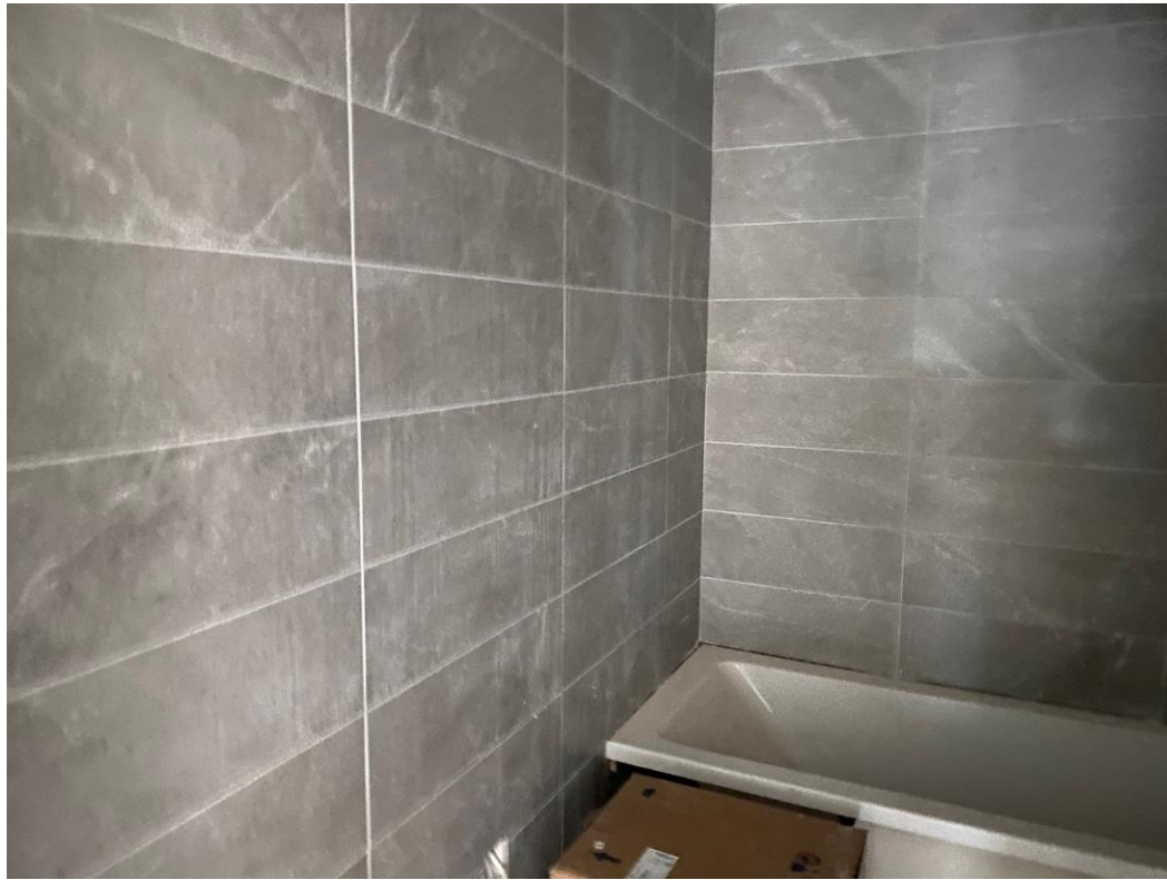
Level 2 – wall and floor tiling
