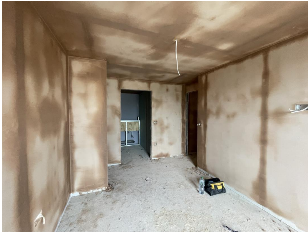
Level 4 – walls and ceilings plastered
