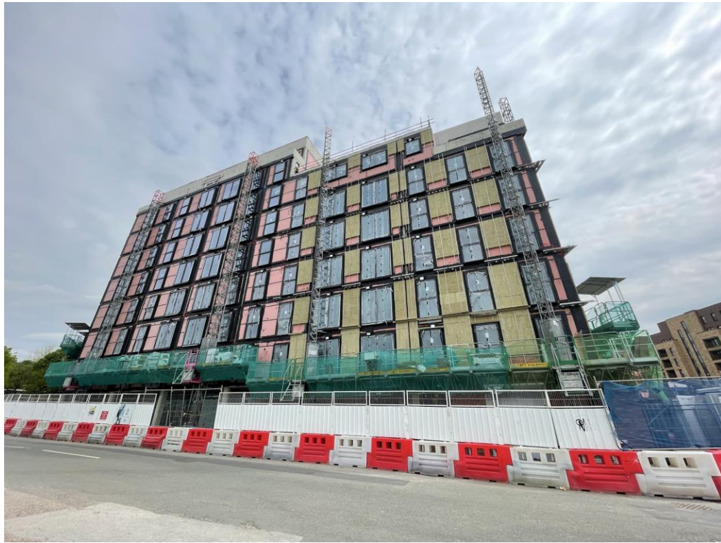
Worrall Street site view
