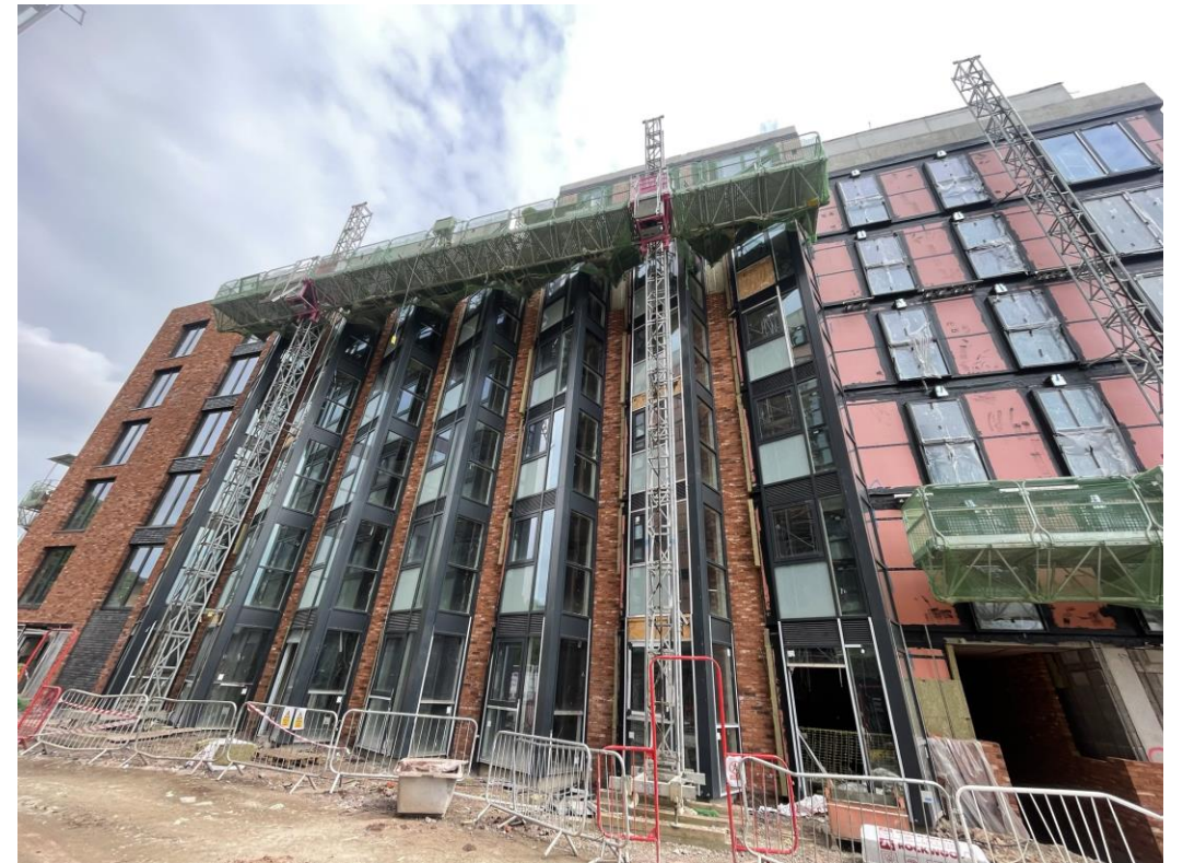
Block B Curtain walling and brickwork
