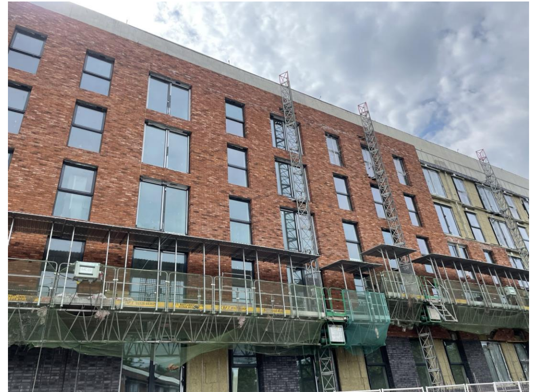
Ordsall Lane site view
