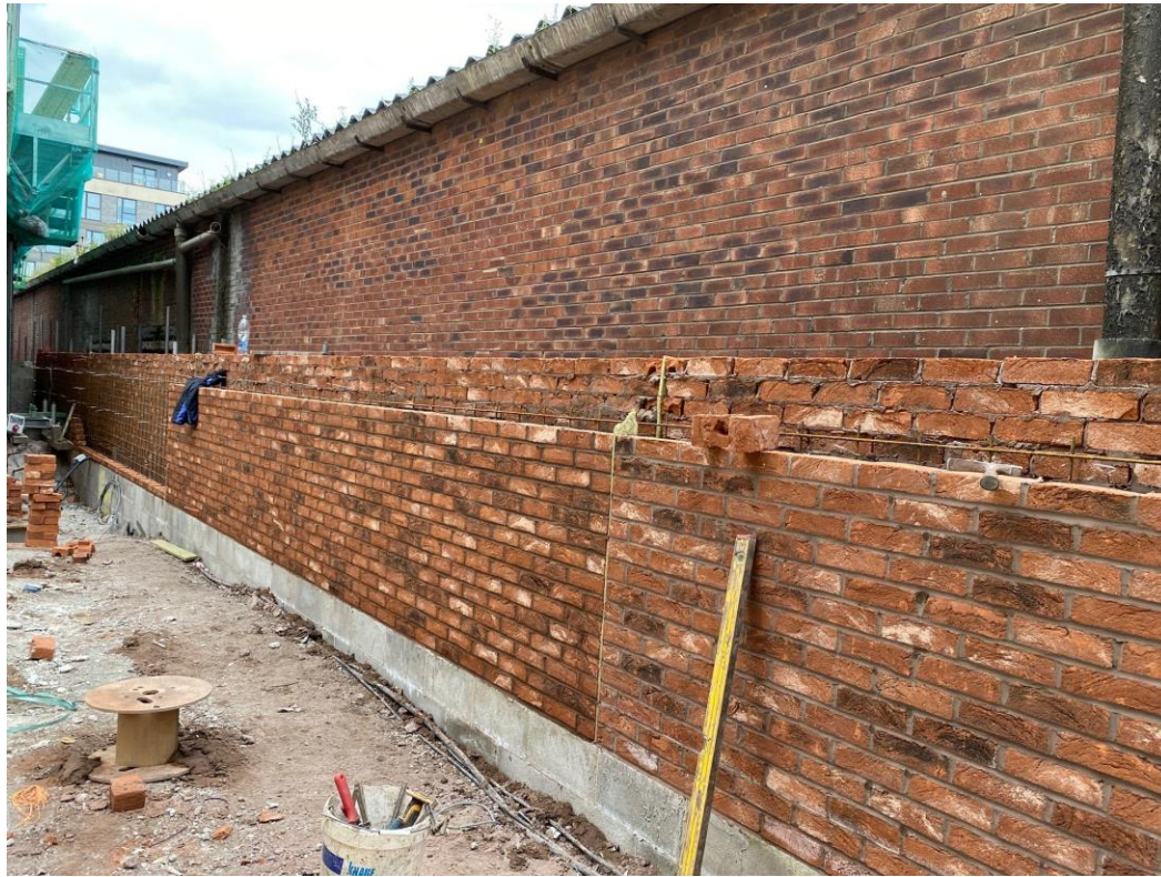
Boundary wall construction
