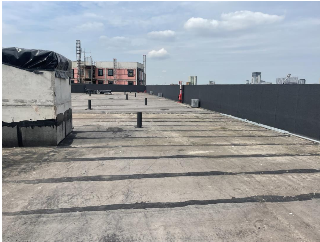
Block B main roof covering preparation
