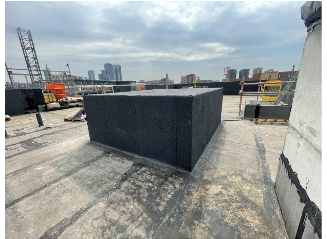
Block B main roof covering preparation
