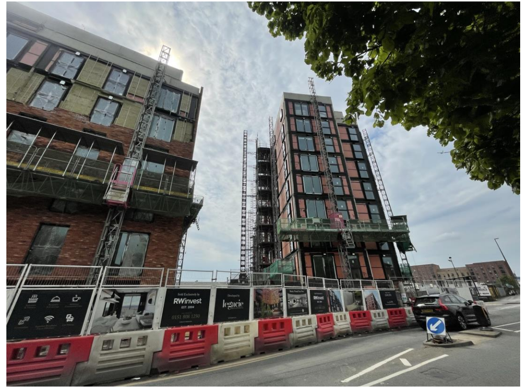
Ordsall Lane site view
