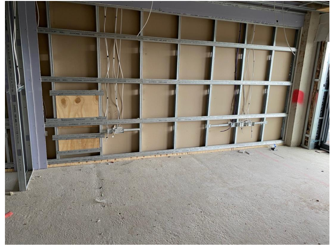
Level 7 – corridor and apartment walls formed
