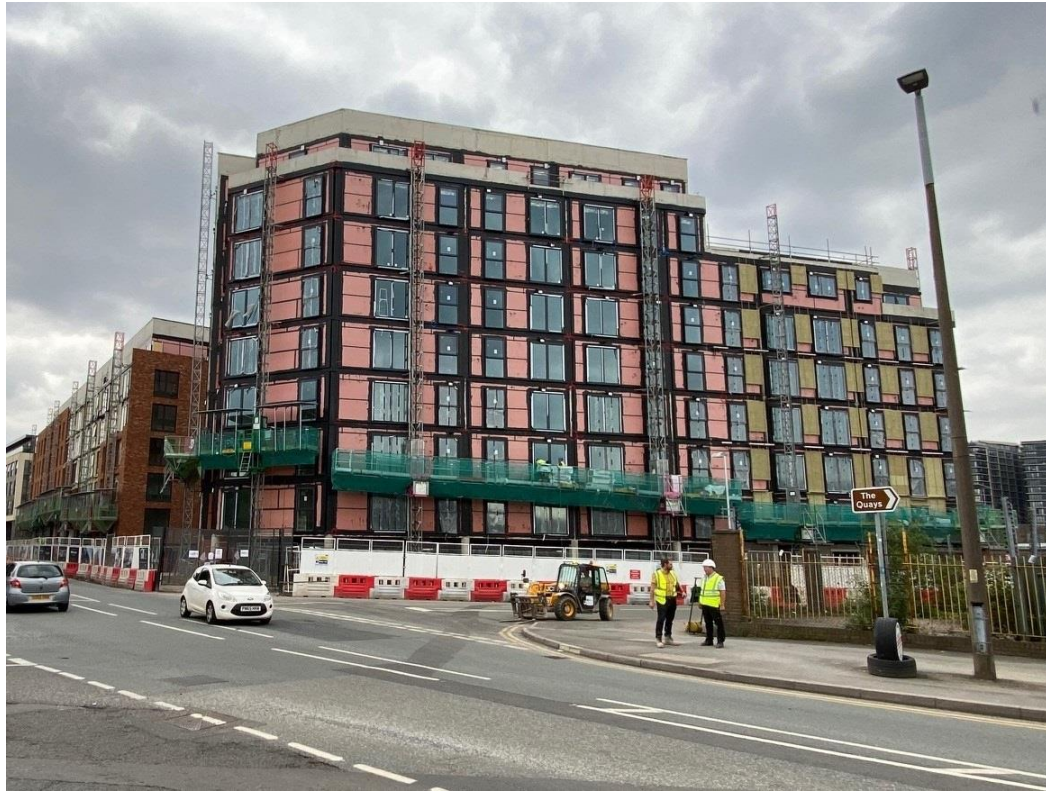
Ordsall Lane site view
