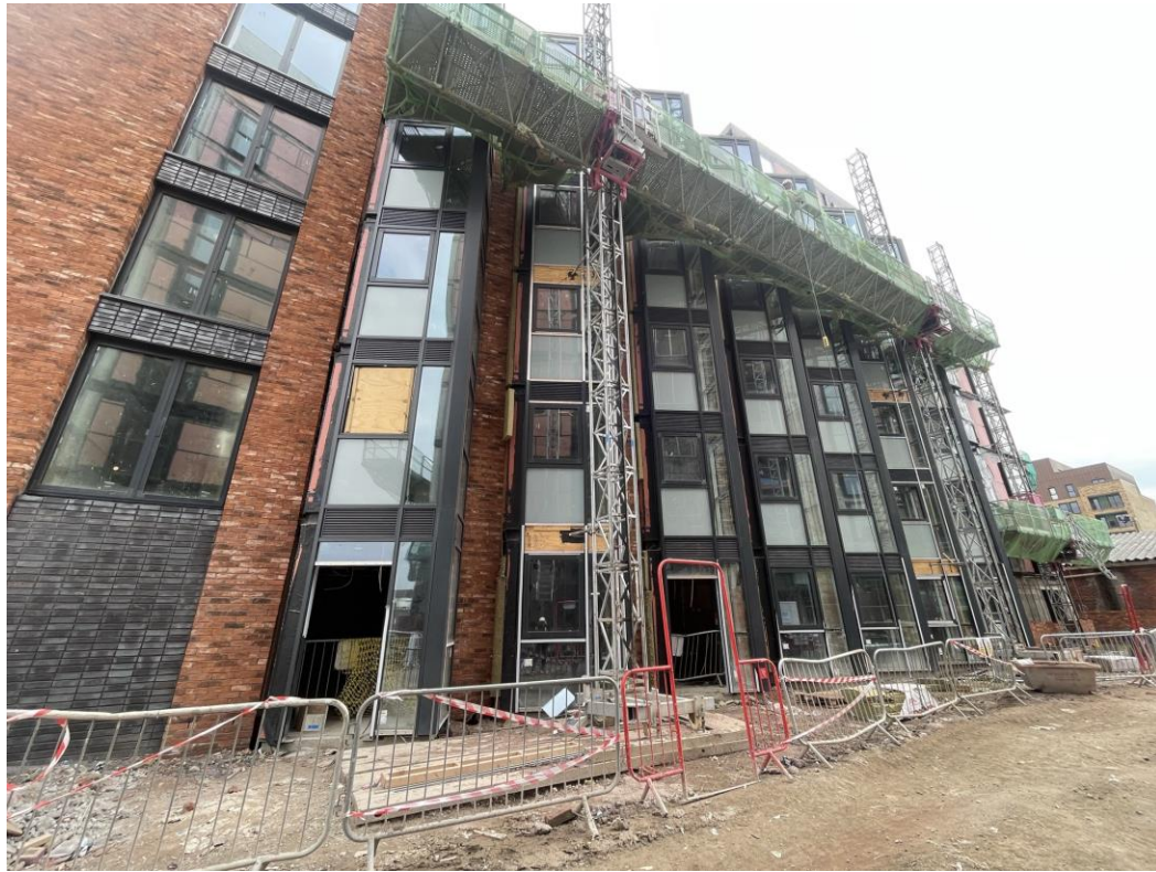
Block B Curtain walling and brickwork
