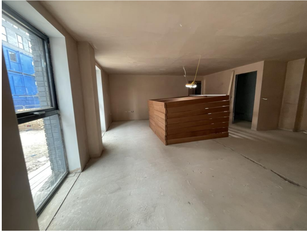
Level 1 – duplex apartment staircase enclosure
