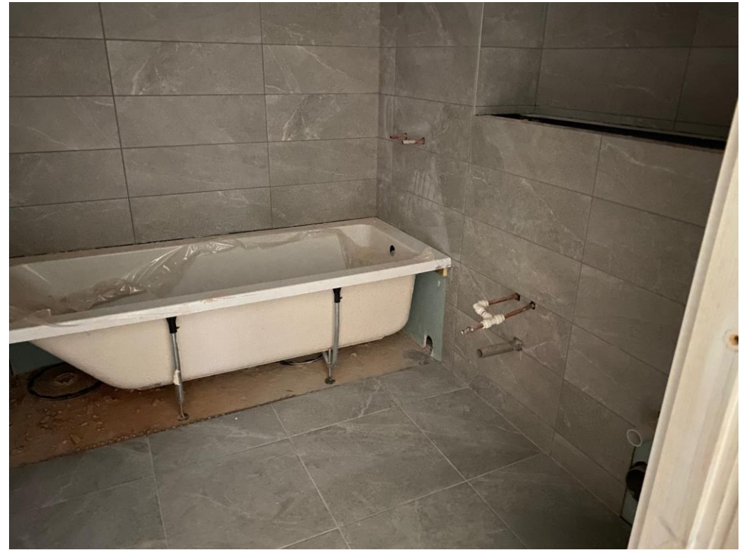
Level 2 – wall and floor tiling
