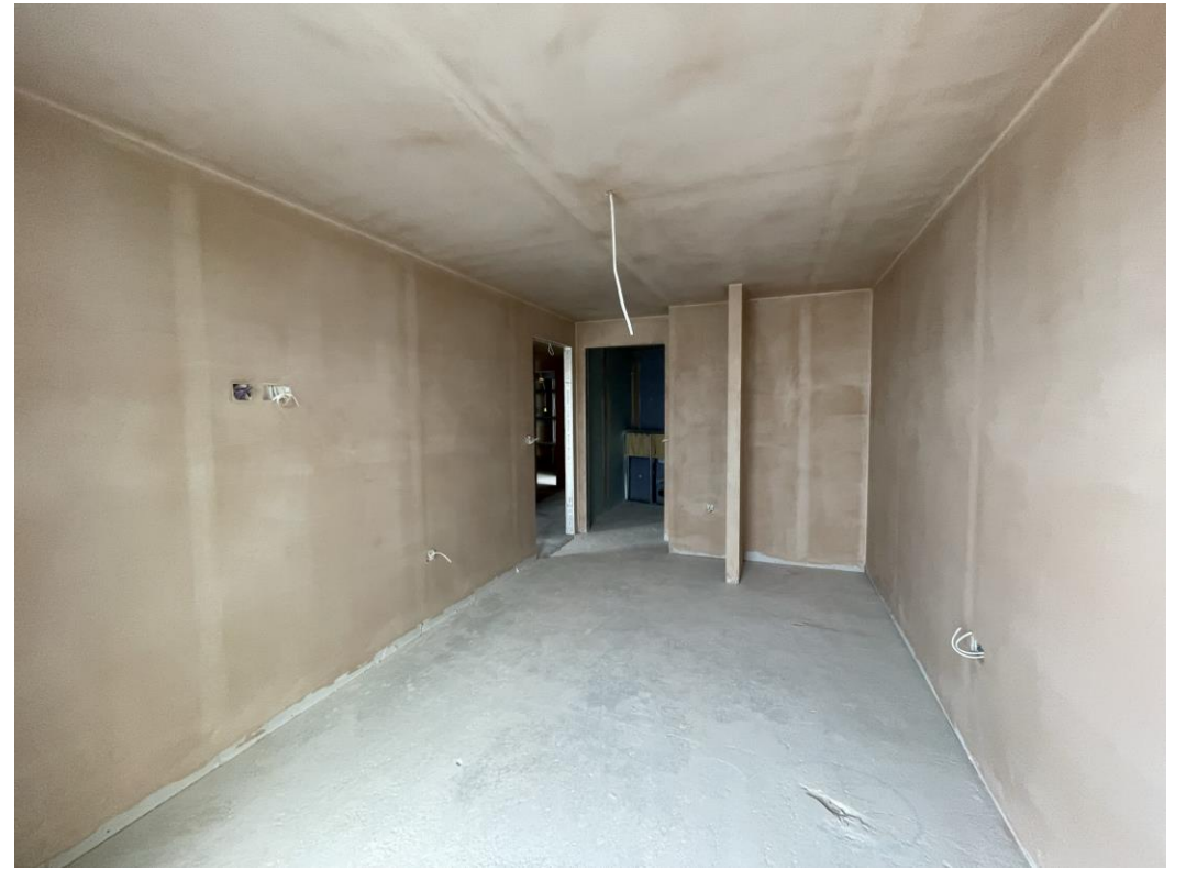
Level 3 – Apartments ready for decoration
