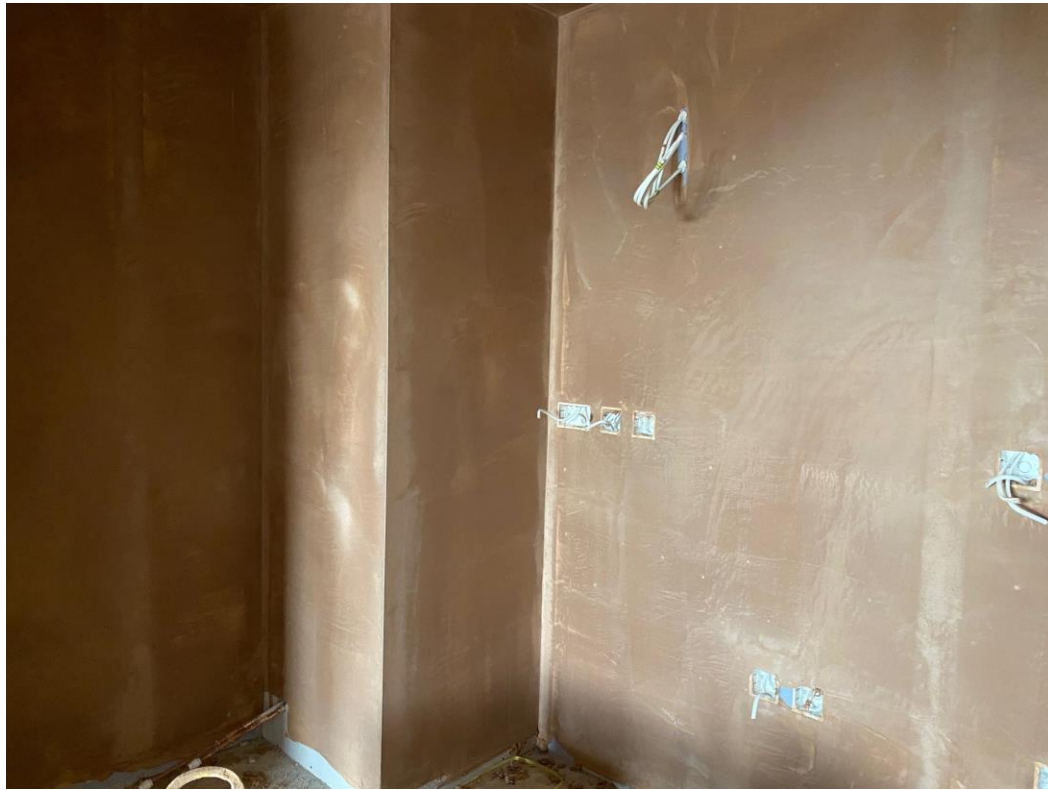
Level 5 – walls and ceilings plastered
