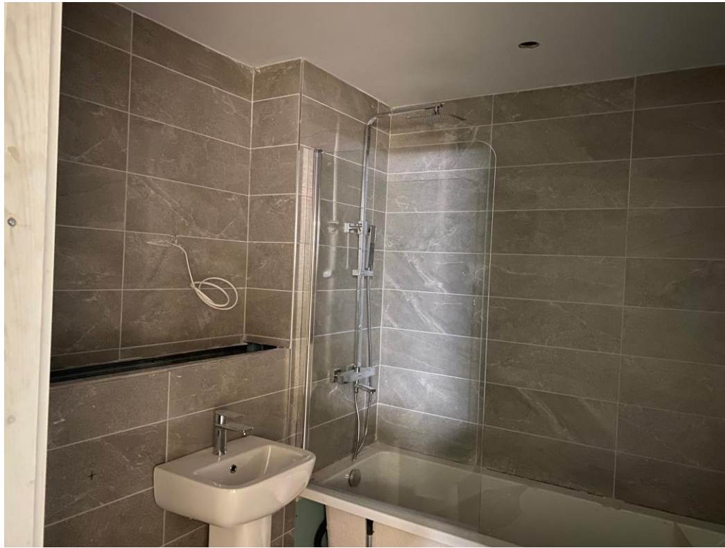
Level 2 – wall and floor tiling
