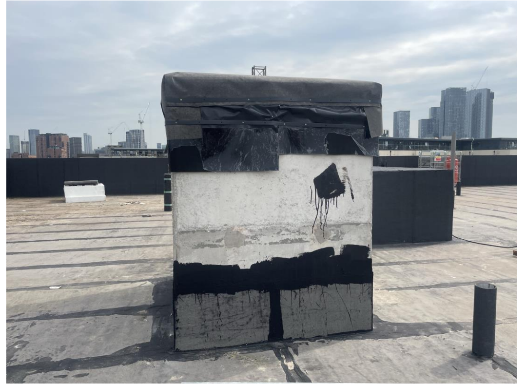
Block B main roof covering preparation
