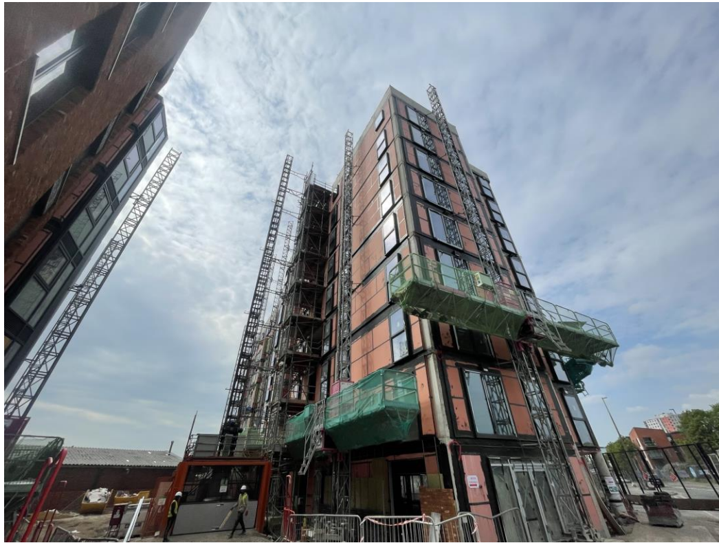
Block A weatherboarding & windows installed
