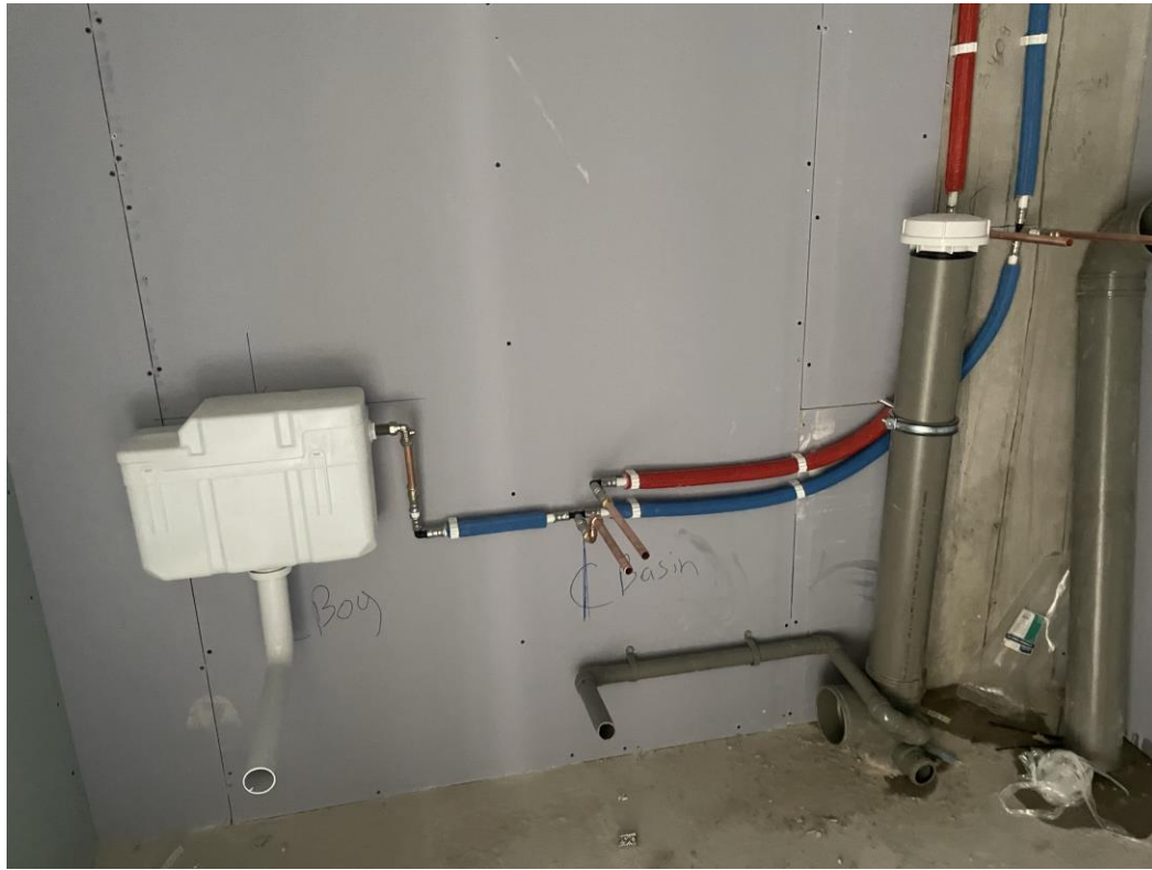
Level 6 – 1 st fix plumbing
