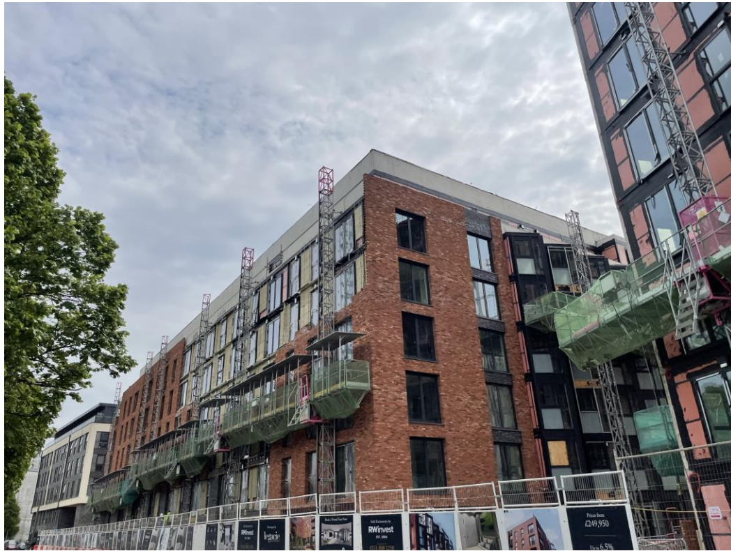
Ordsall Lane site view
