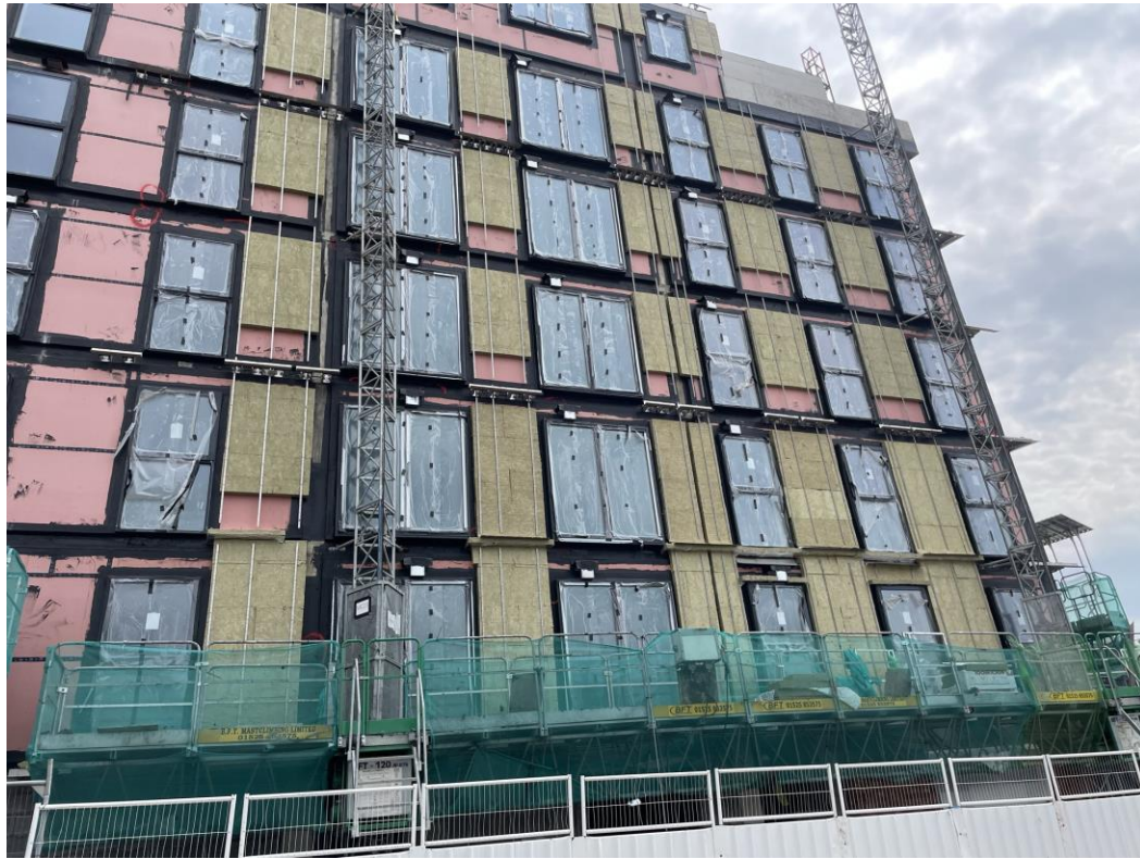
Worrall Street site view
