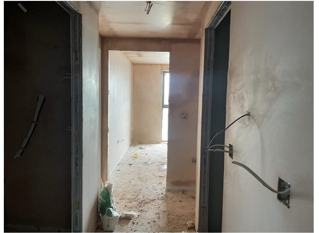
Level 4 – walls and ceilings plastered
