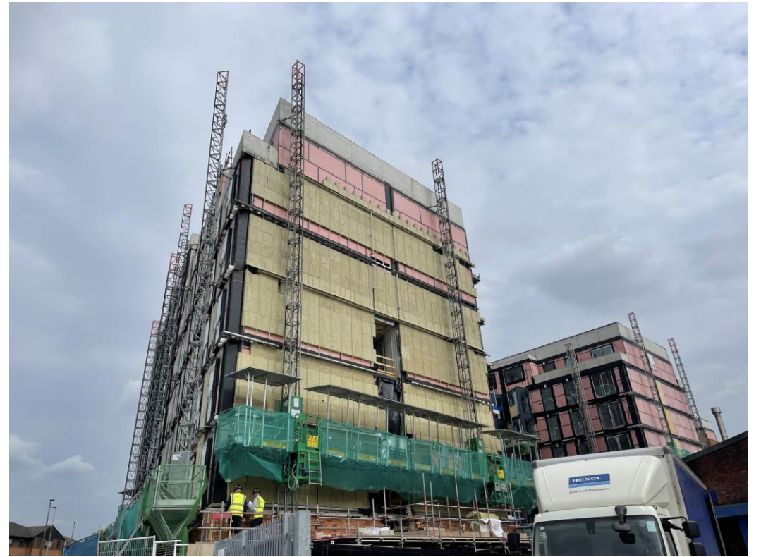
Worrall Street site view
