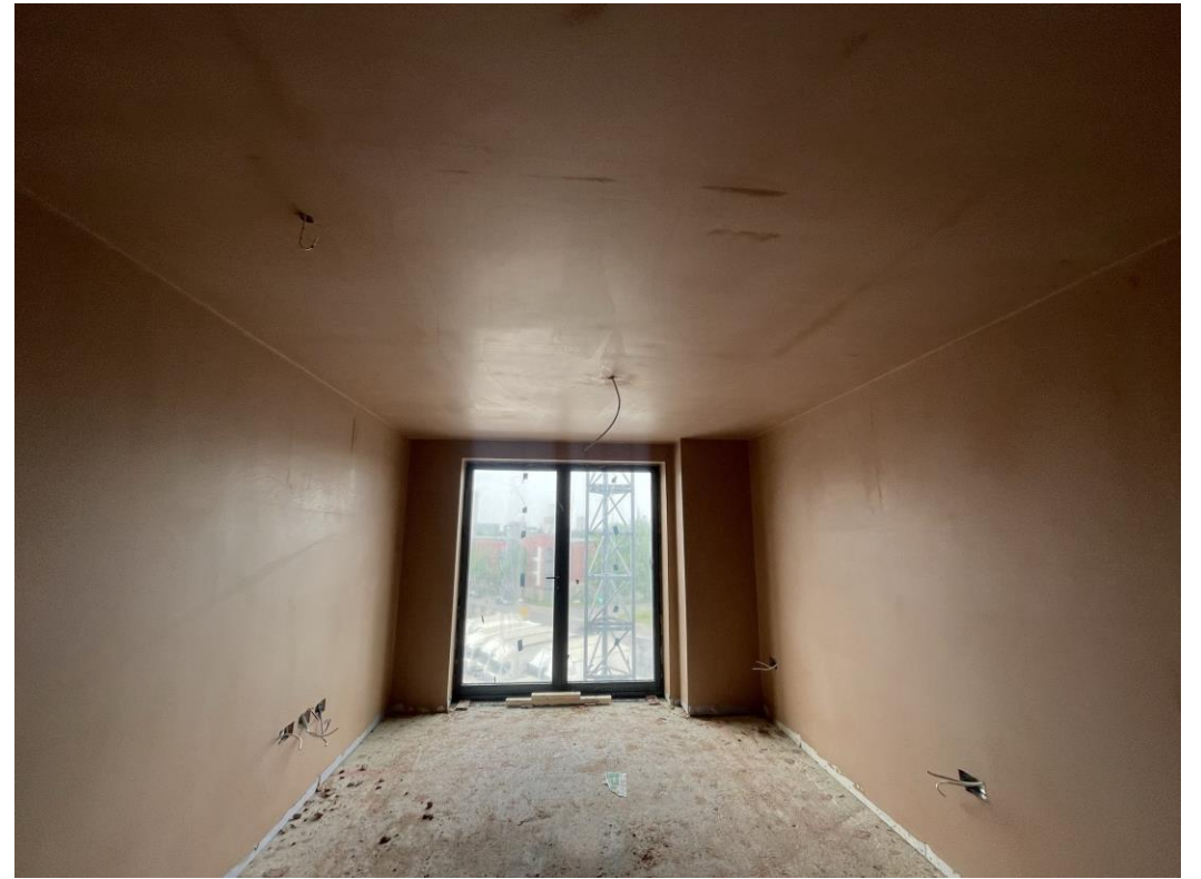
Level 4 – walls and ceilings plastered
