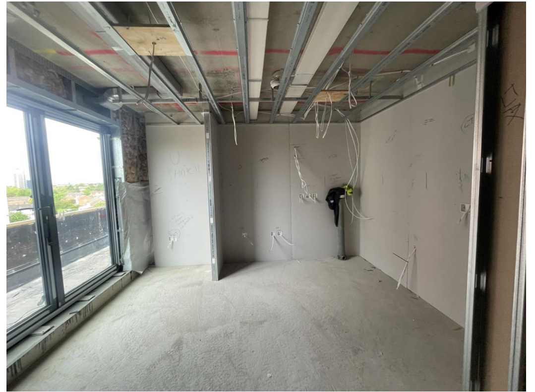
Level 6 – corridor and apartment walls formed
