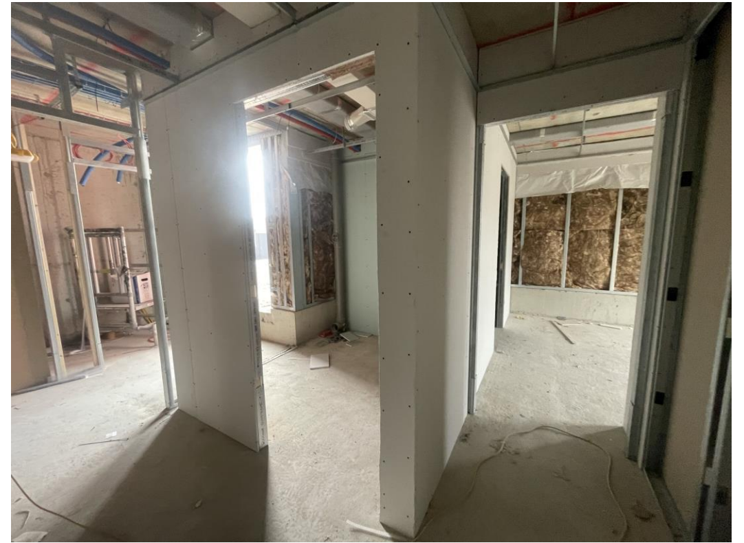
Level 7 – corridor and apartment walls formed
