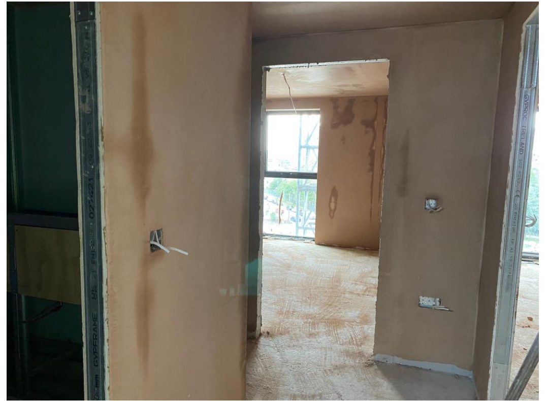
Level 5 – walls and ceilings plastered
