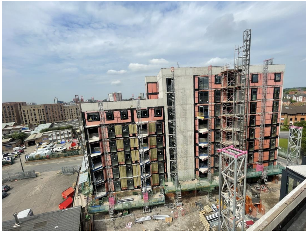
Block A weatherboarding & windows installed
