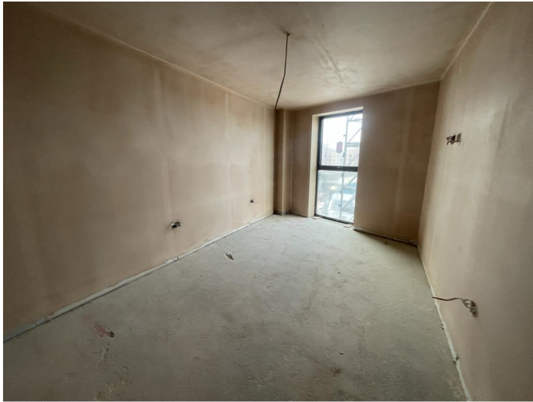
Level 3 – Apartments ready for decoration
