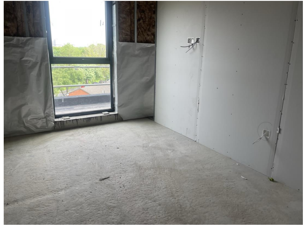
Level 6 – corridor and apartment walls formed
