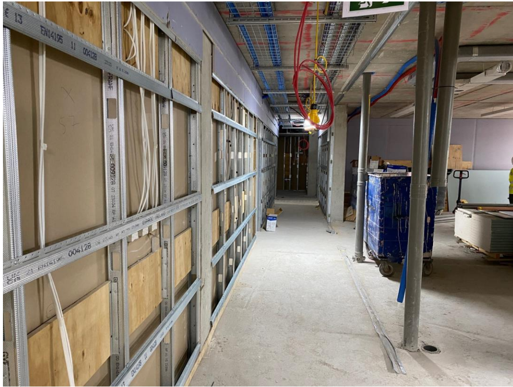
Level 7 – corridor and apartment walls formed
