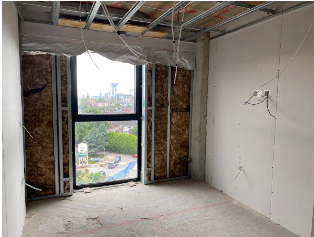
Level 7 – corridor and apartment walls formed
