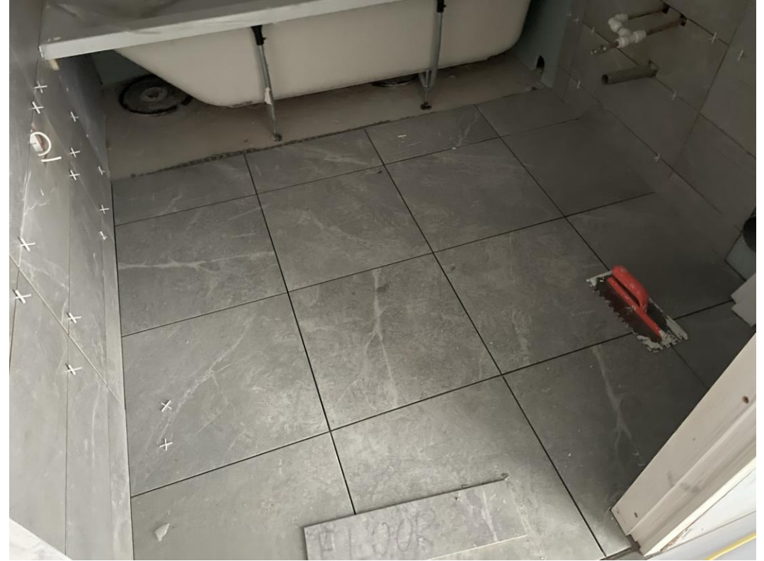
Level 1 – Apartment wall & floor tiling
