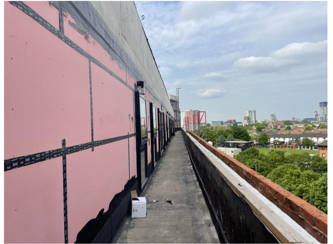
Block B parapet brickwork
