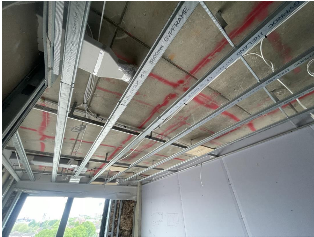
Level 6 – suspended ceiling installation
