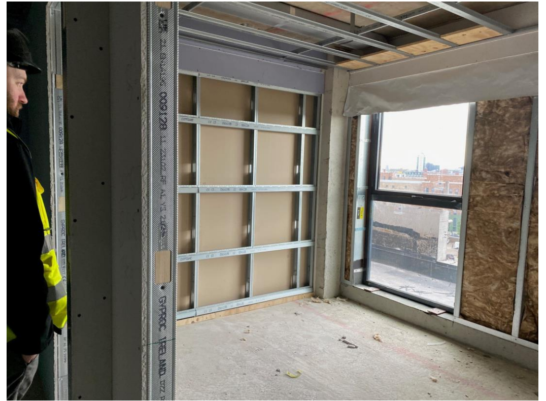
Level 8 – corridor and apartment walls formed
