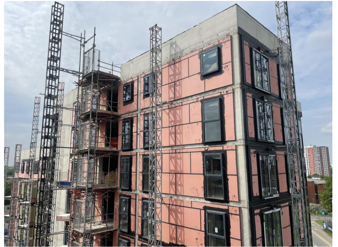
Block A weatherboarding & windows installed
