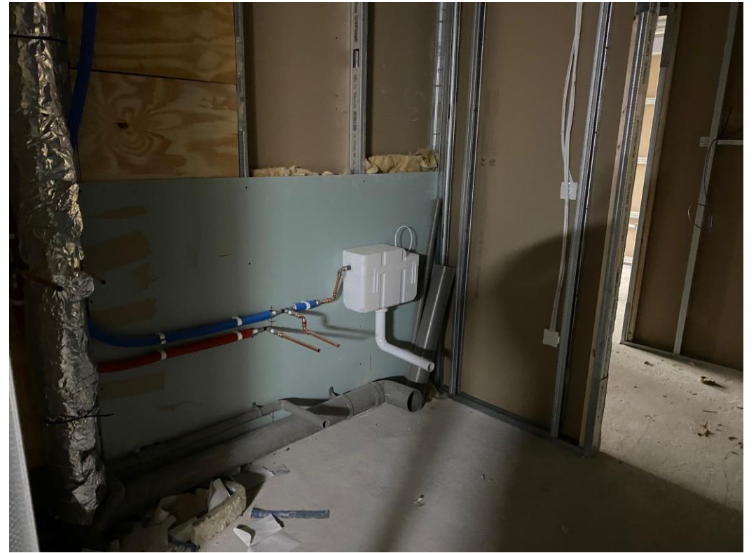
Level 6 – 1 st fix plumbing
