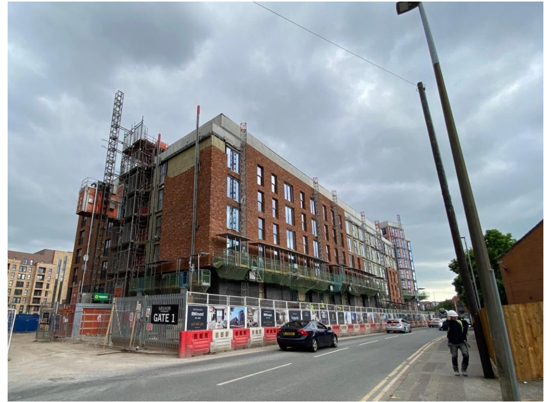
Ordsall Lane site view
