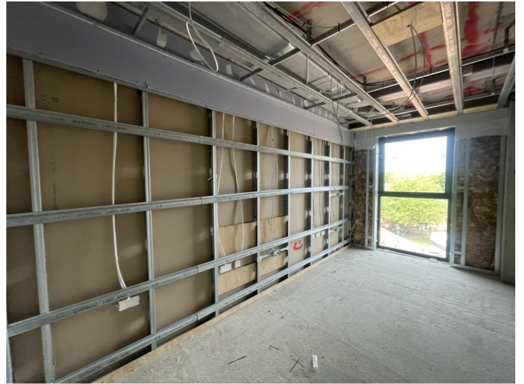
Level 5 – corridor and apartment walls formed
