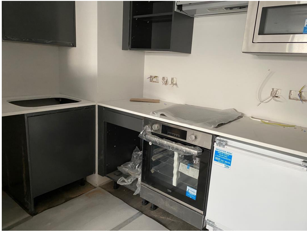
Level 1 – Kitchen installed
