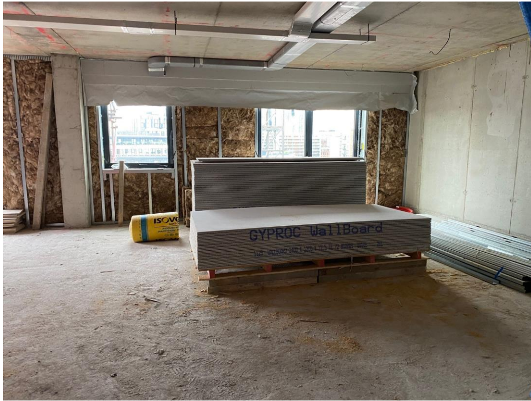
Level 8 – corridor and apartment walls formed
