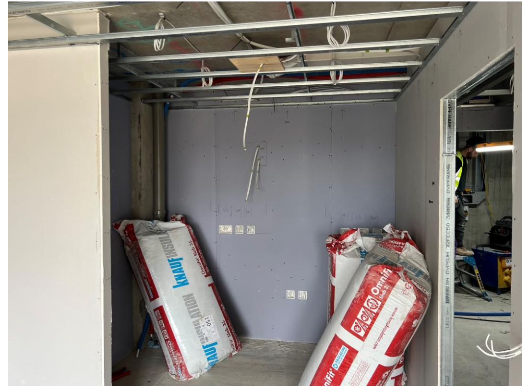
Level 5 – ceiling installation
