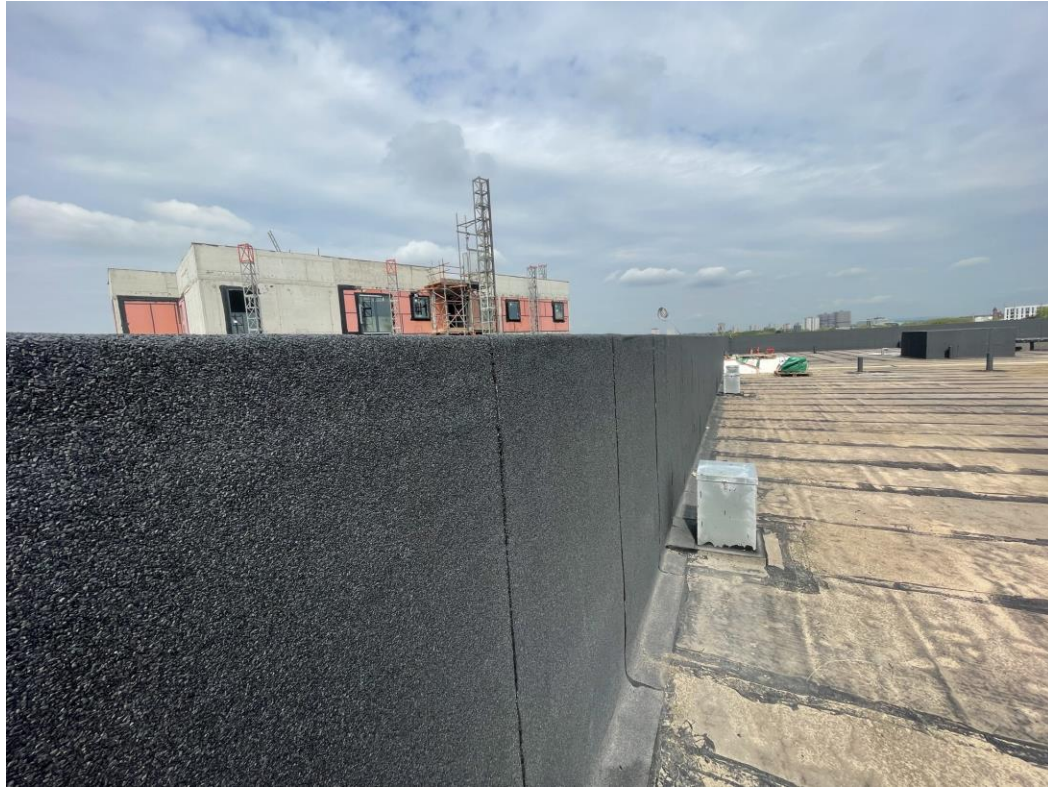
Block B main roof covering preparation
