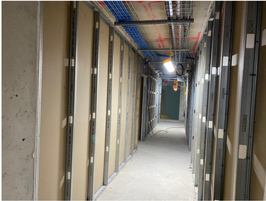
Level 8 – corridor and apartment walls formed
