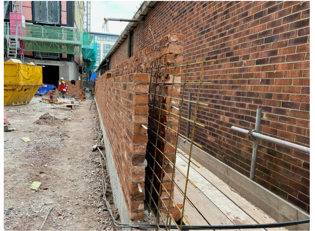
Boundary wall construction
