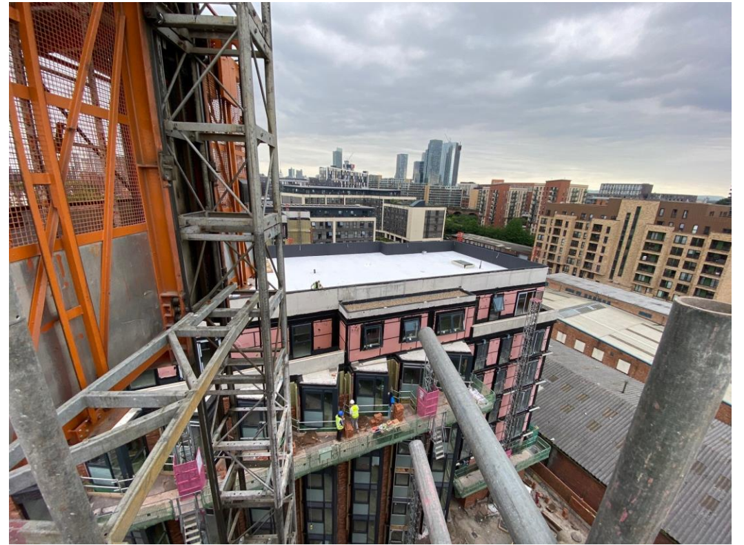
Block B main roof covering preparation
