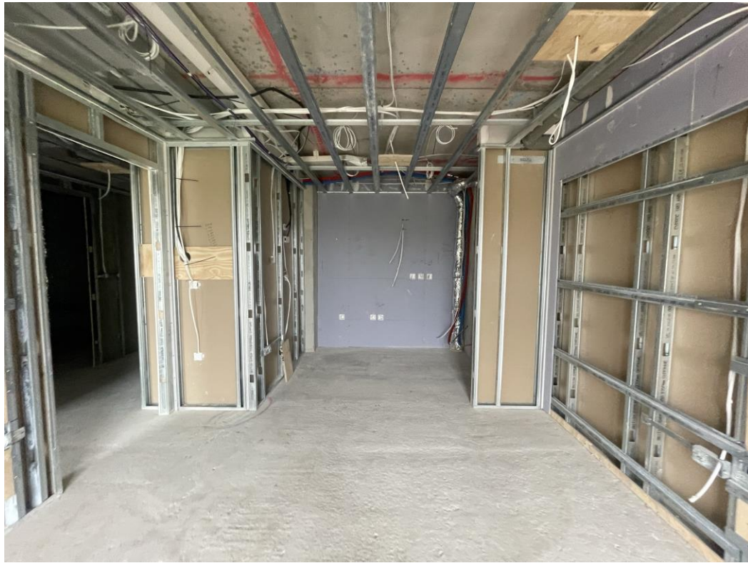
Level 5 – corridor and apartment walls formed
