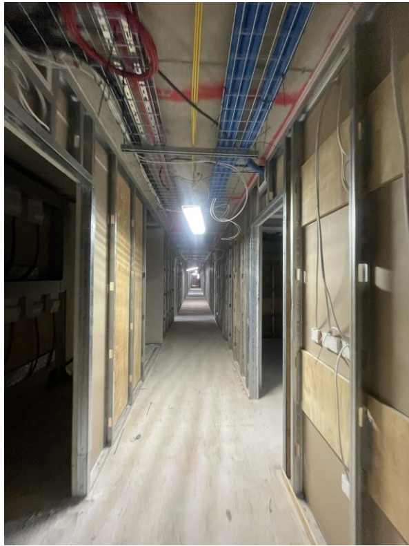
Level 5 – corridor and apartment walls formed
