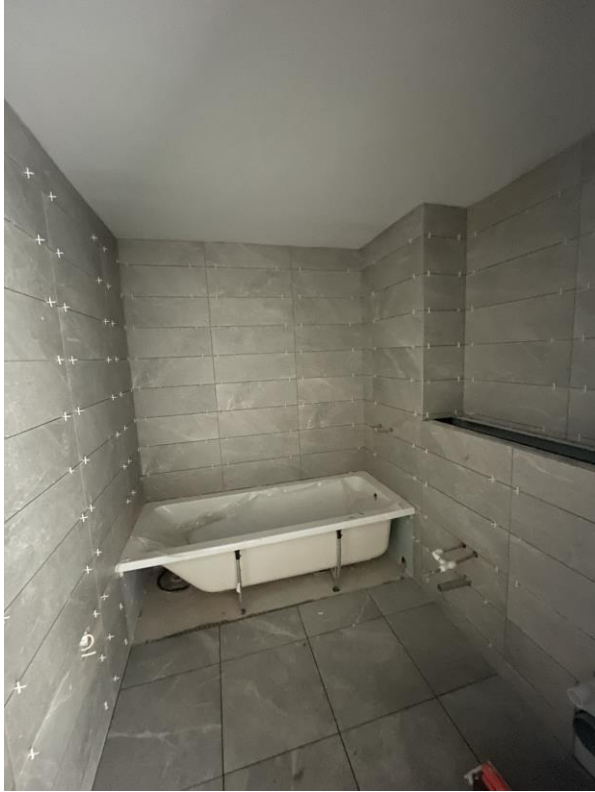
Level 1 – Apartment wall & floor tiling
