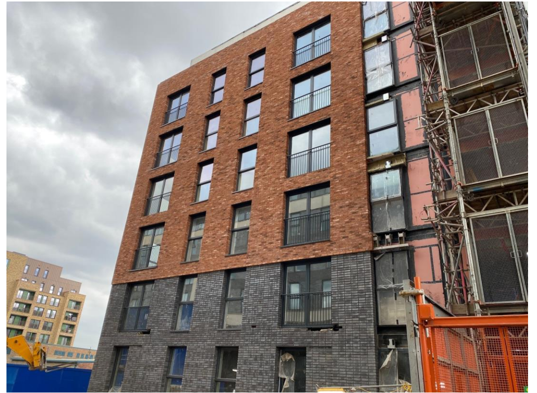
Ordsall Lane site view
