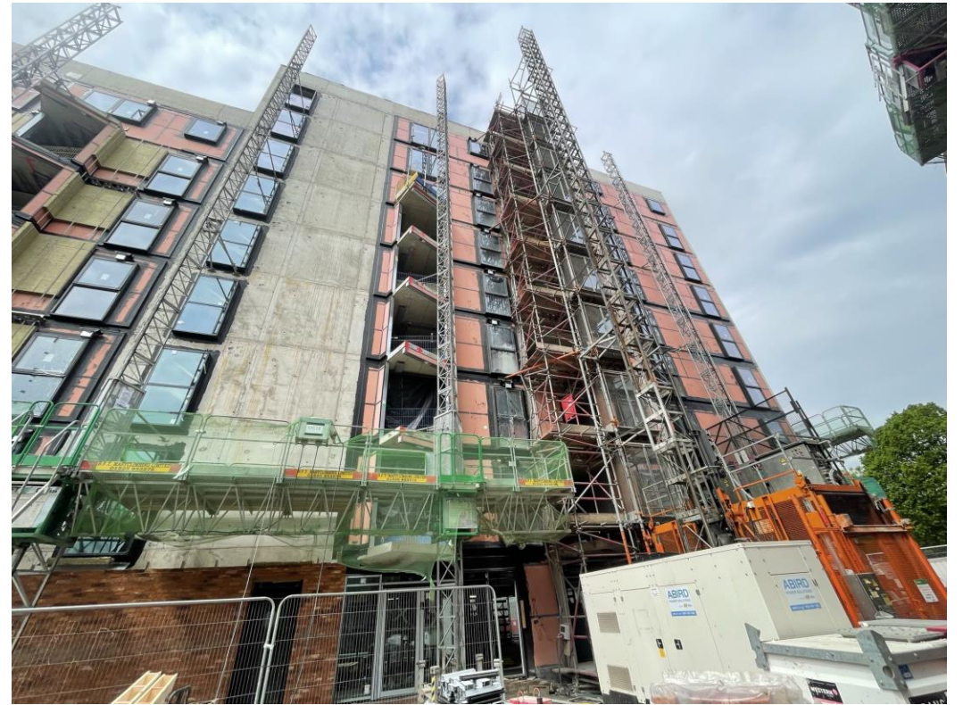
Block A weatherboarding & windows installed
