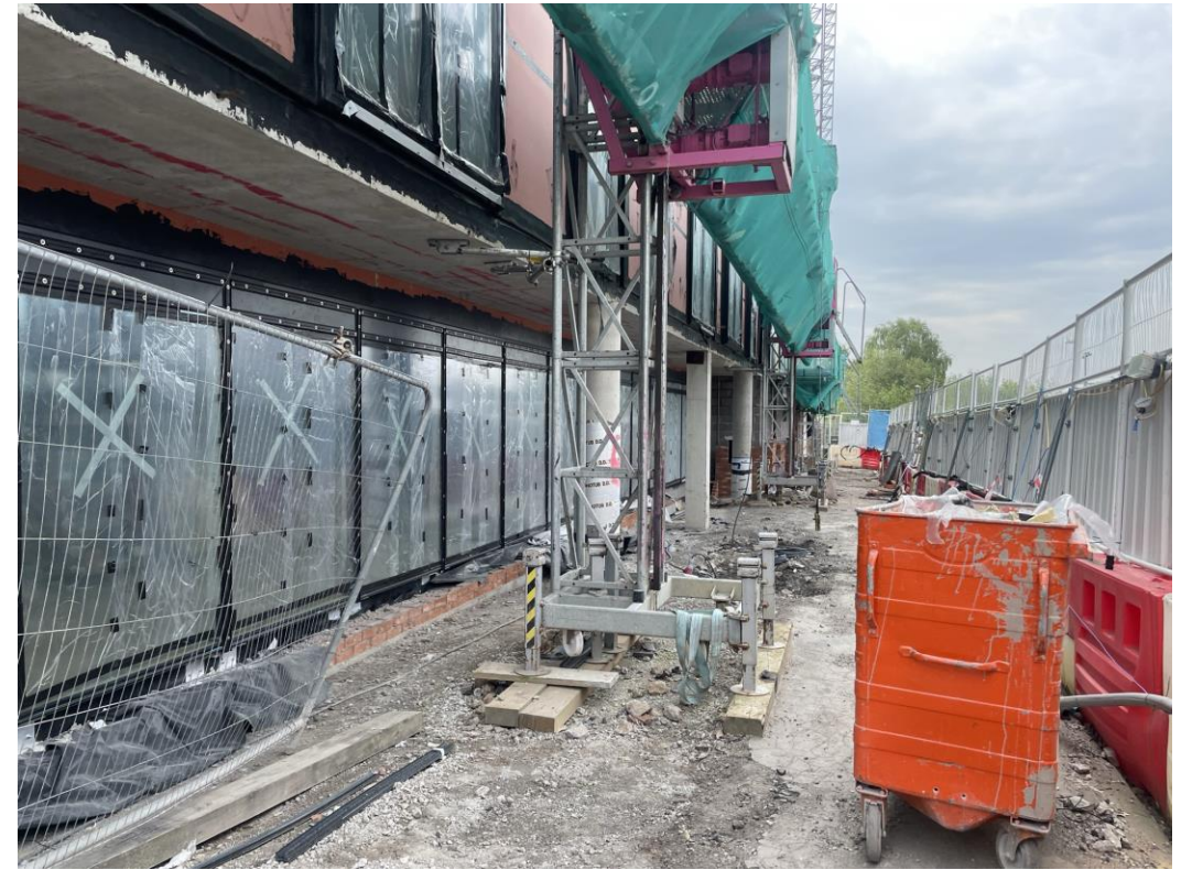
Block A weatherboarding & windows installed
