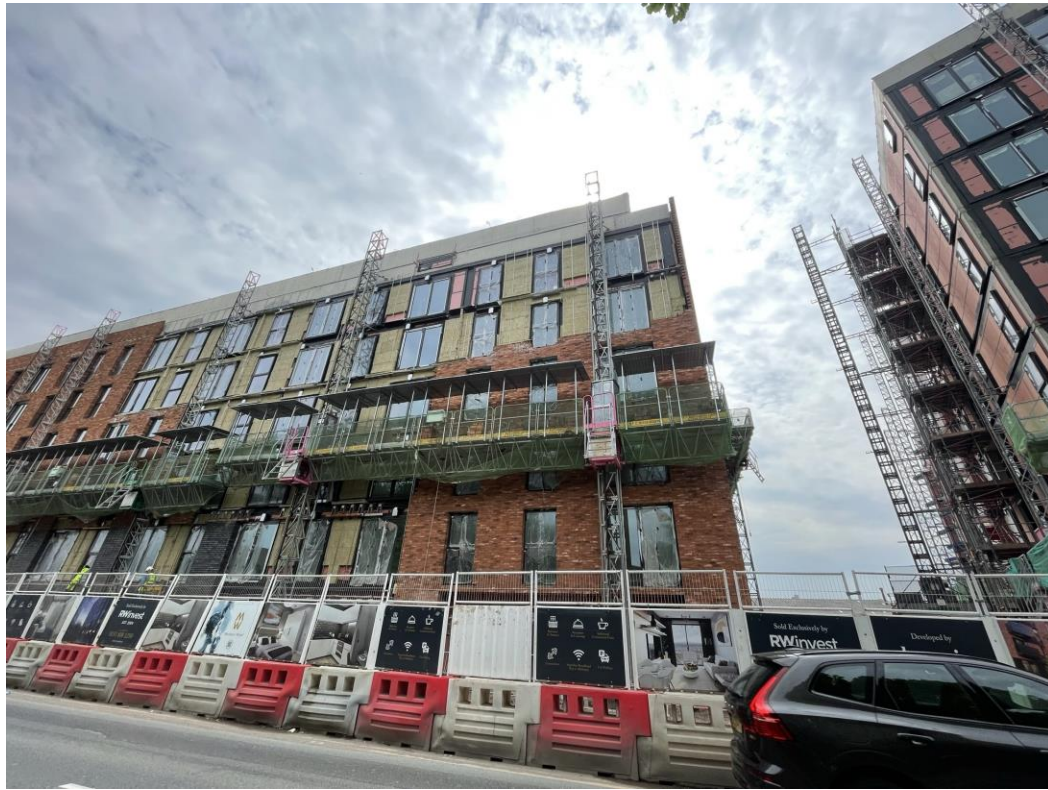
Ordsall Lane site view
