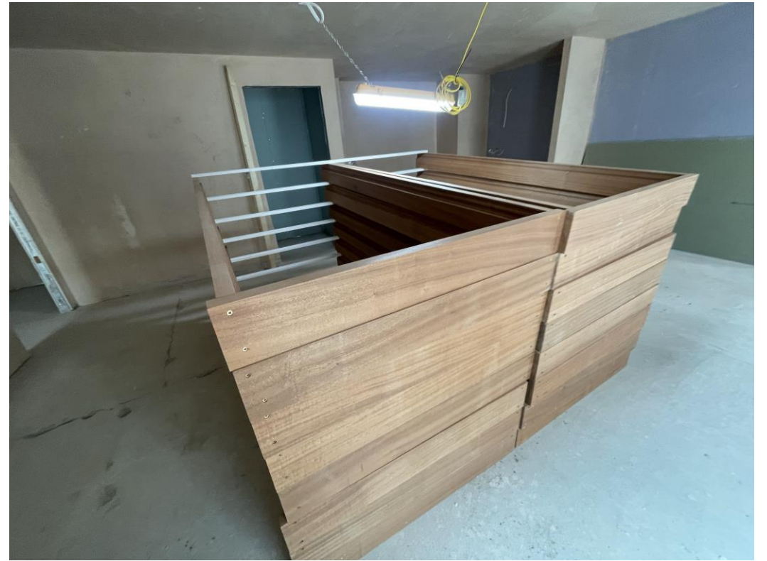
Level 1 – duplex apartment staircase enclosure
