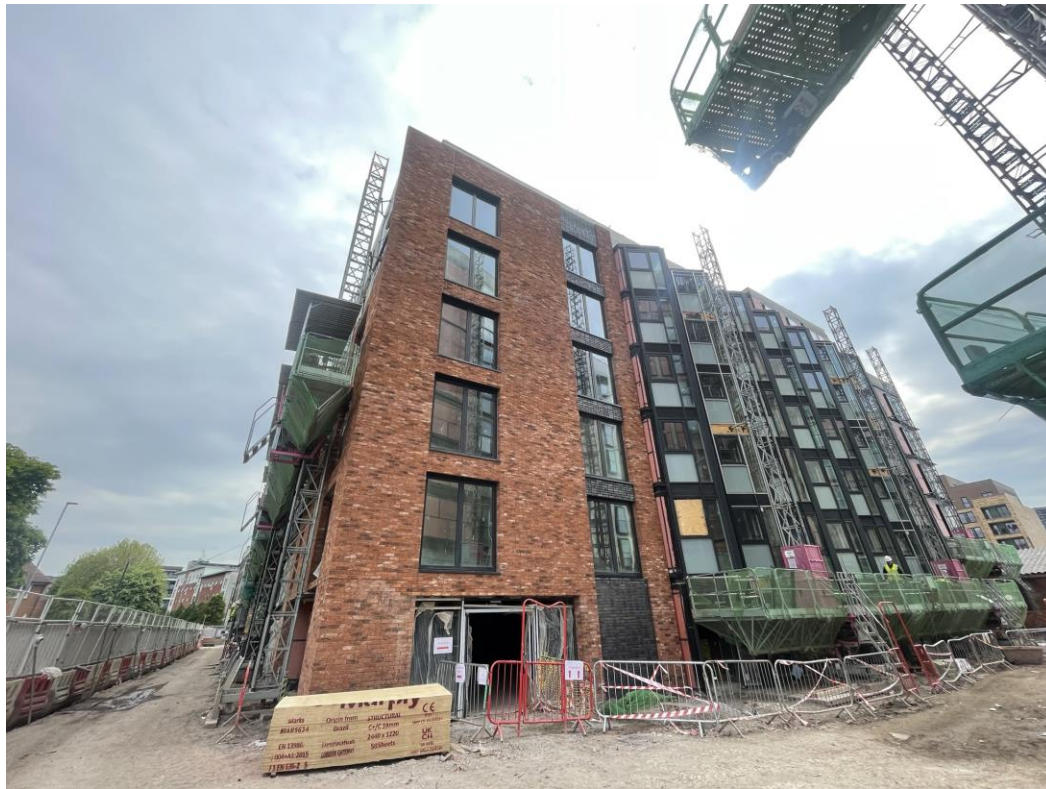
Block B Curtain walling and brickwork
