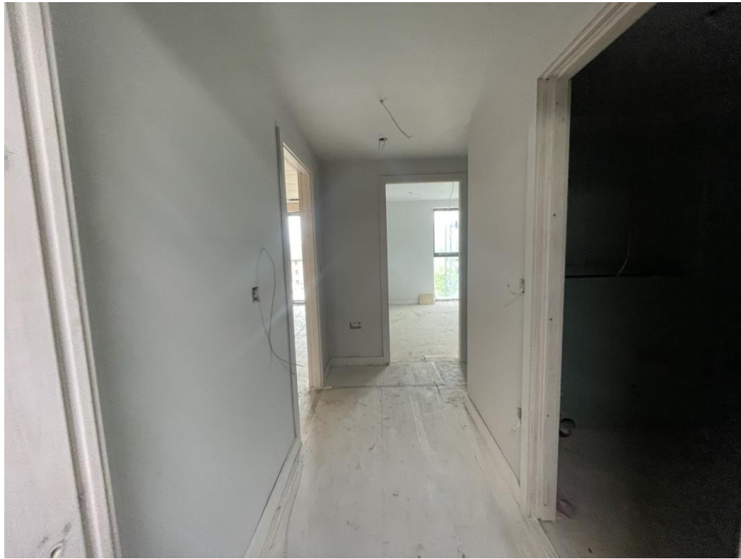
Level 4 – doorframes, skirting & architrave
