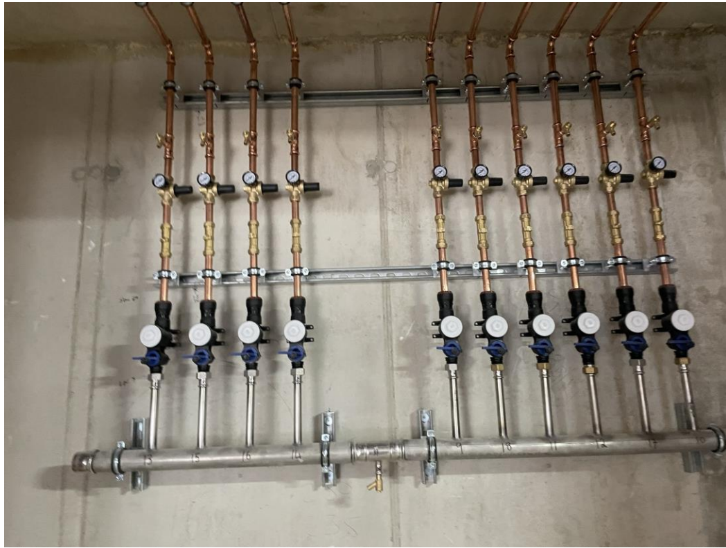
Level 3 – mains water services connections
