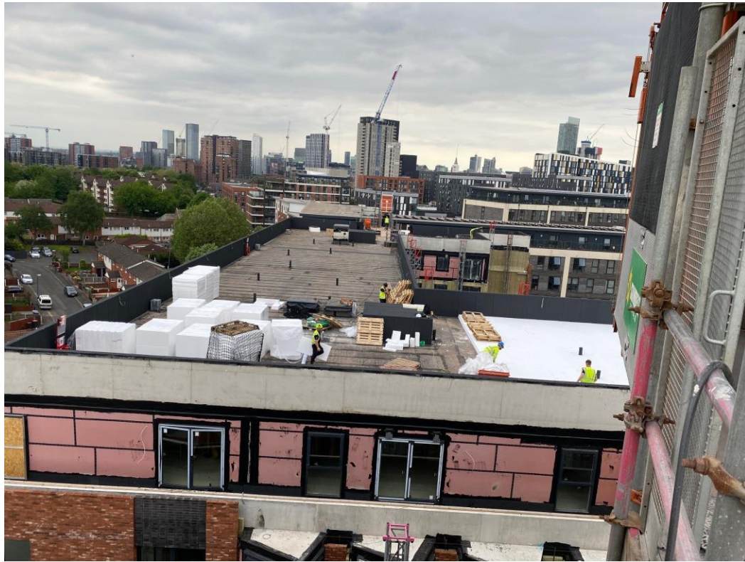
Block B main roof covering preparation
