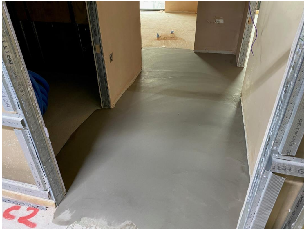
Level 3 – Apartments ready for decoration
