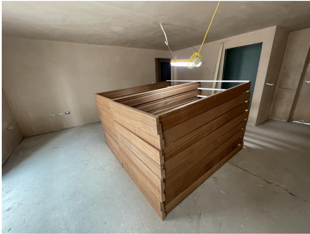
Level 1 – duplex apartment staircase enclosure
