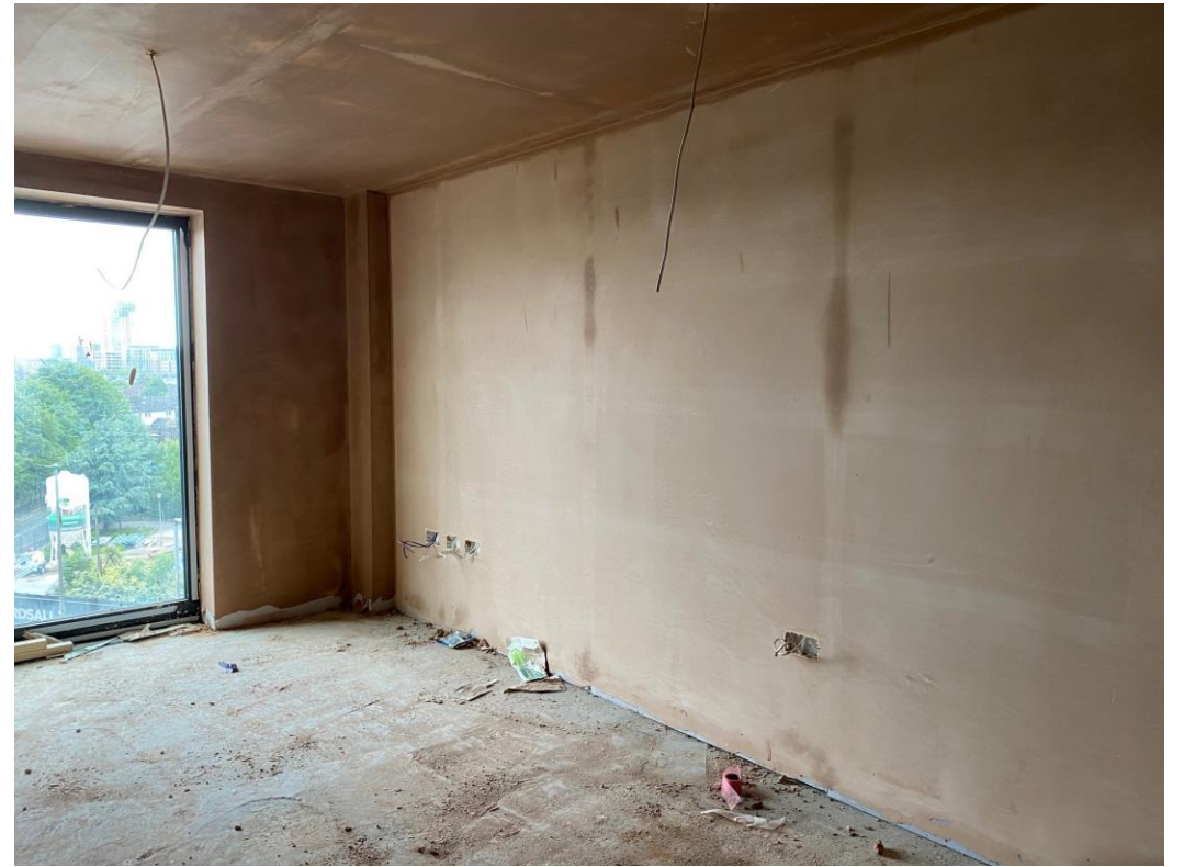
Level 5 – walls and ceilings plastered
