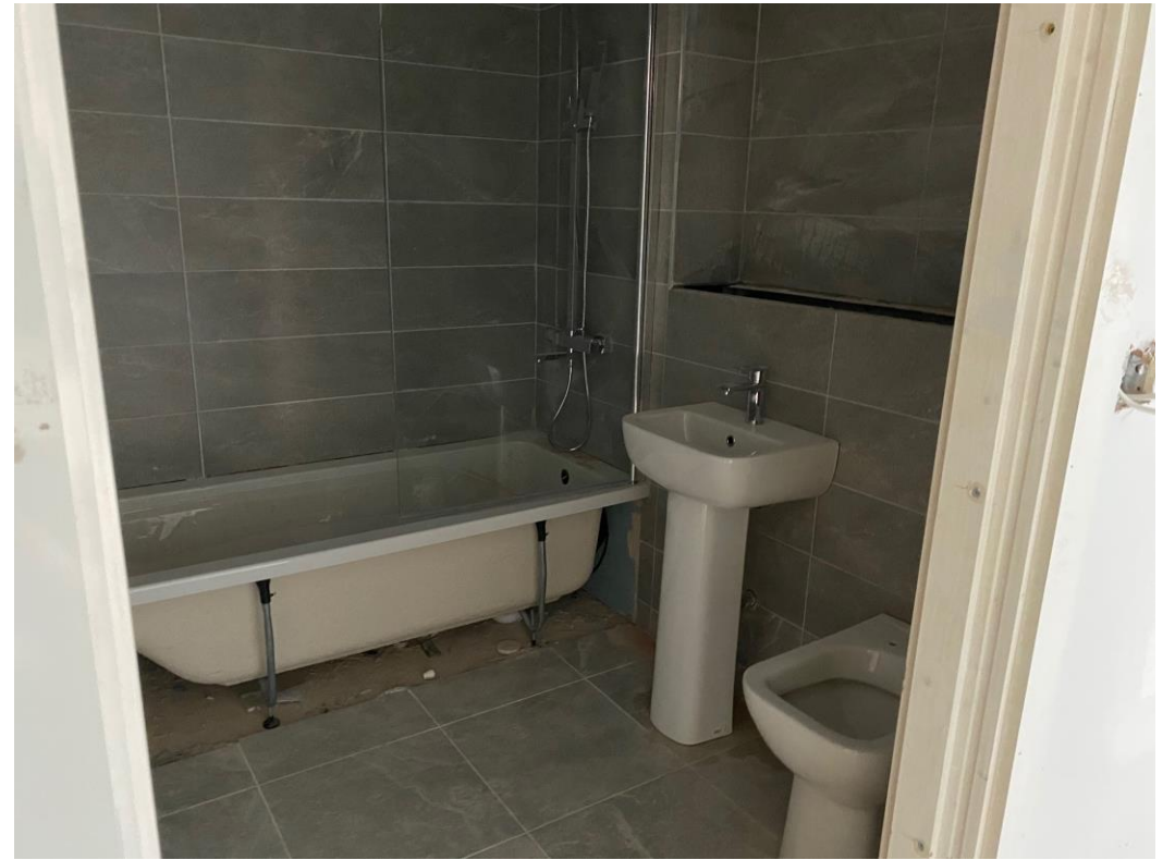
Level 2 – wall and floor tiling
