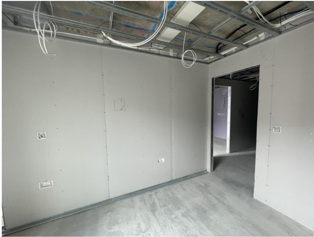
Level 5 – walls boarded
