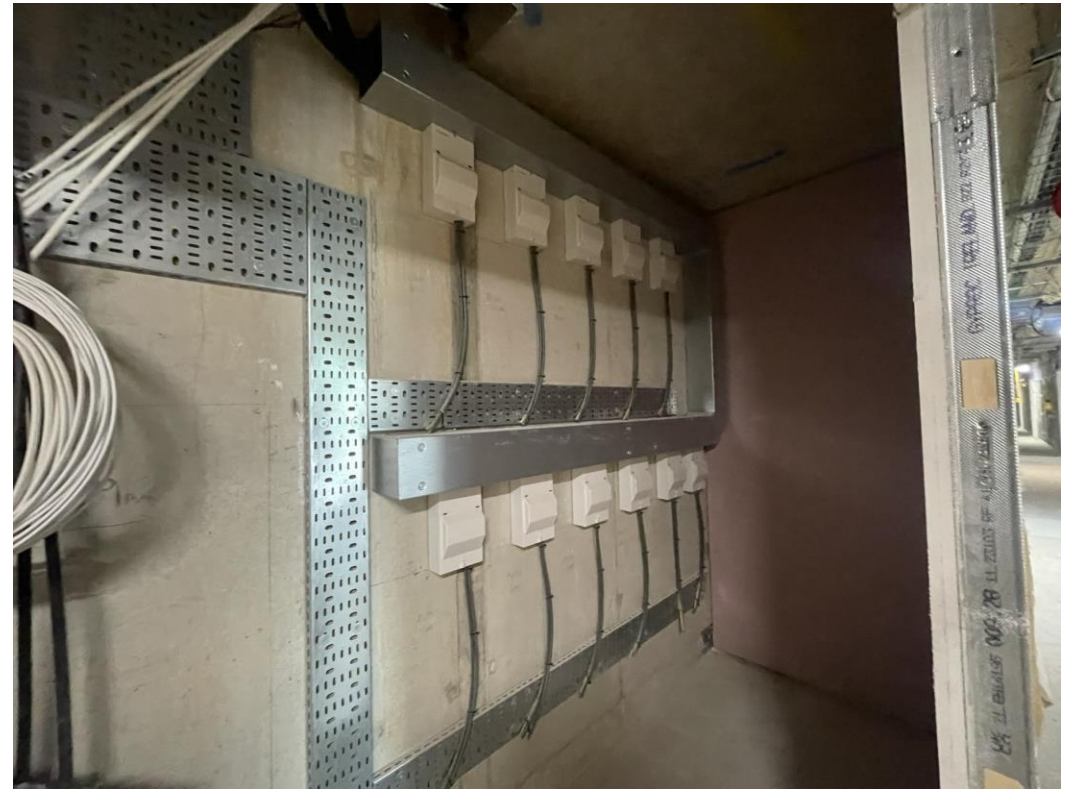
Level 3 – electrical mains services connections
