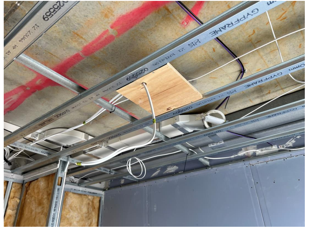
Level 4 – 1 st fix electrical
