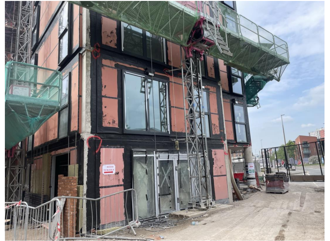
Block A weatherboarding & windows installed
