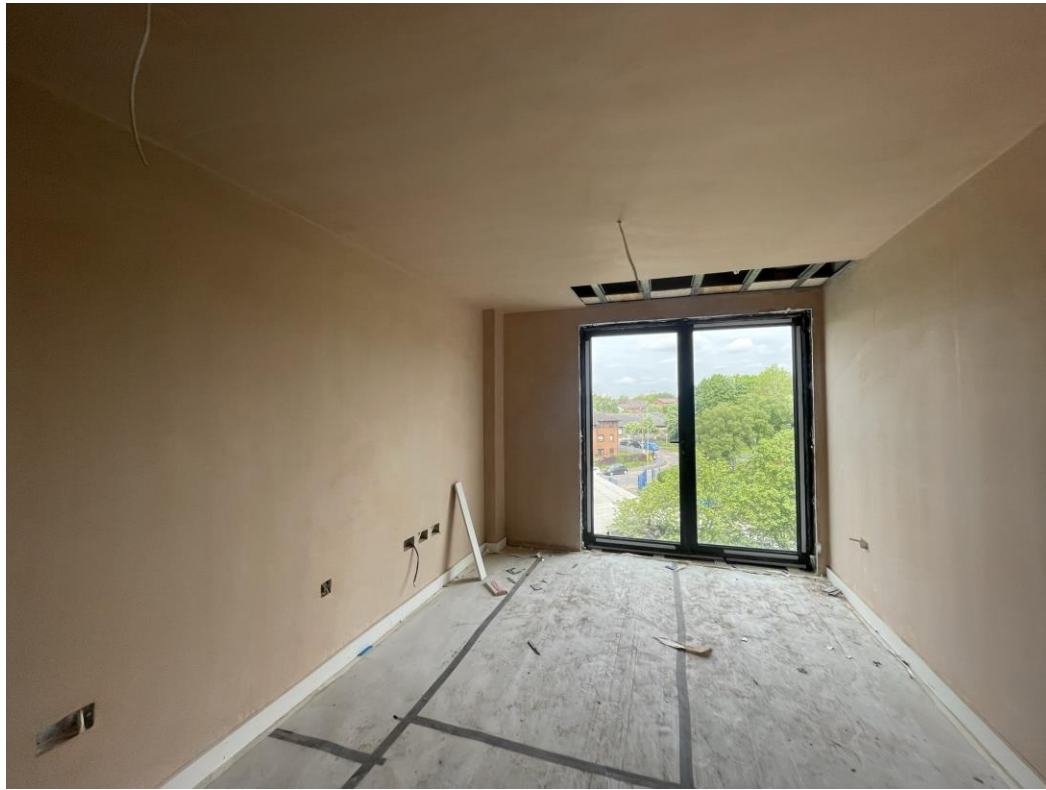
Level 4 - apartments plastered
