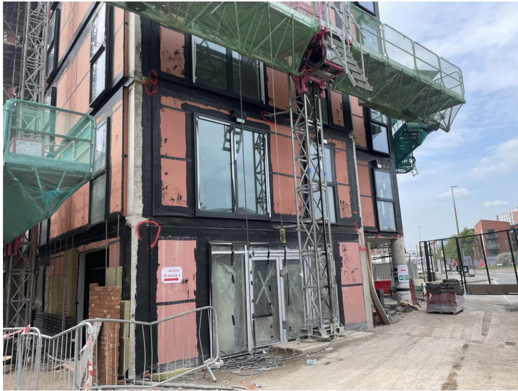
Block A weatherboarding & windows installed
