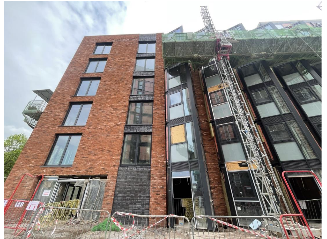
Block B Curtain walling and brickwork
