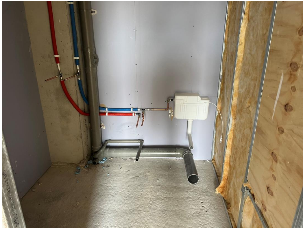
Level 5 – 1 st fix plumbing
