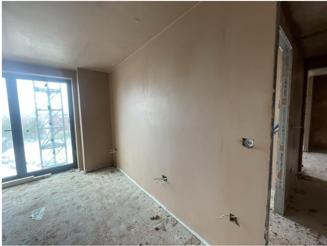
Level 4 – walls and ceilings plastered
