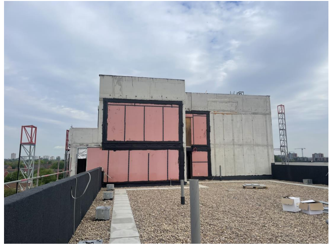
Block A inverted terrace roof system complete
