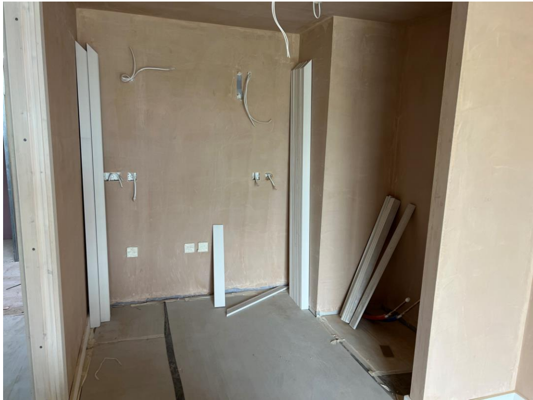
Upper floor apartments plastered
