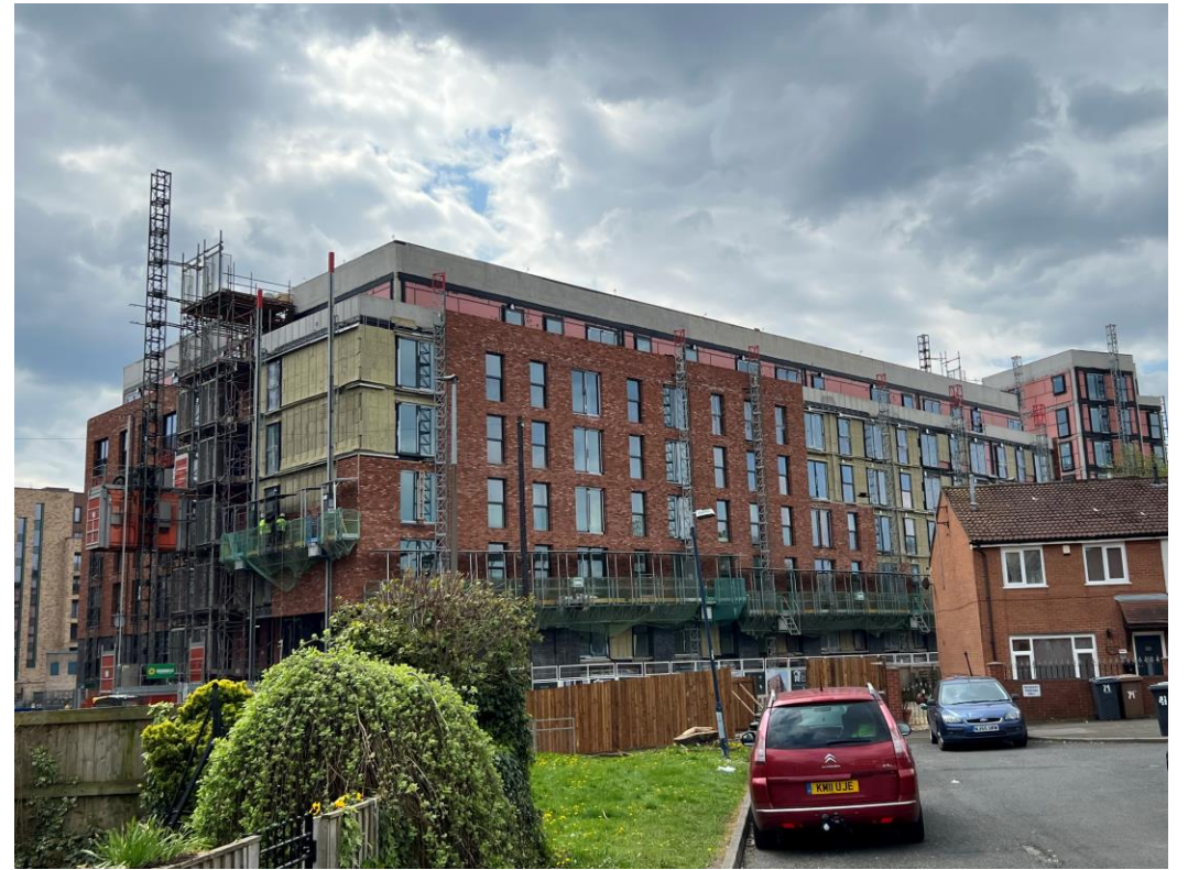
Ordsall Lane site view
