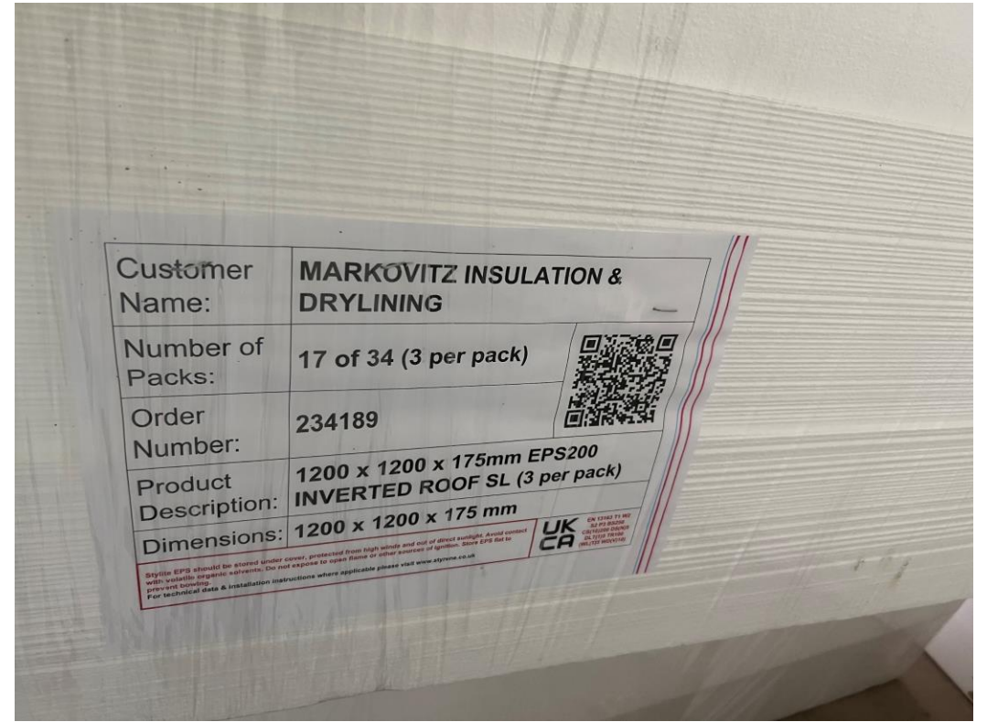
Block A roof insulation stored
