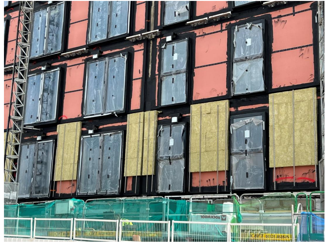
Worrall Street site view
