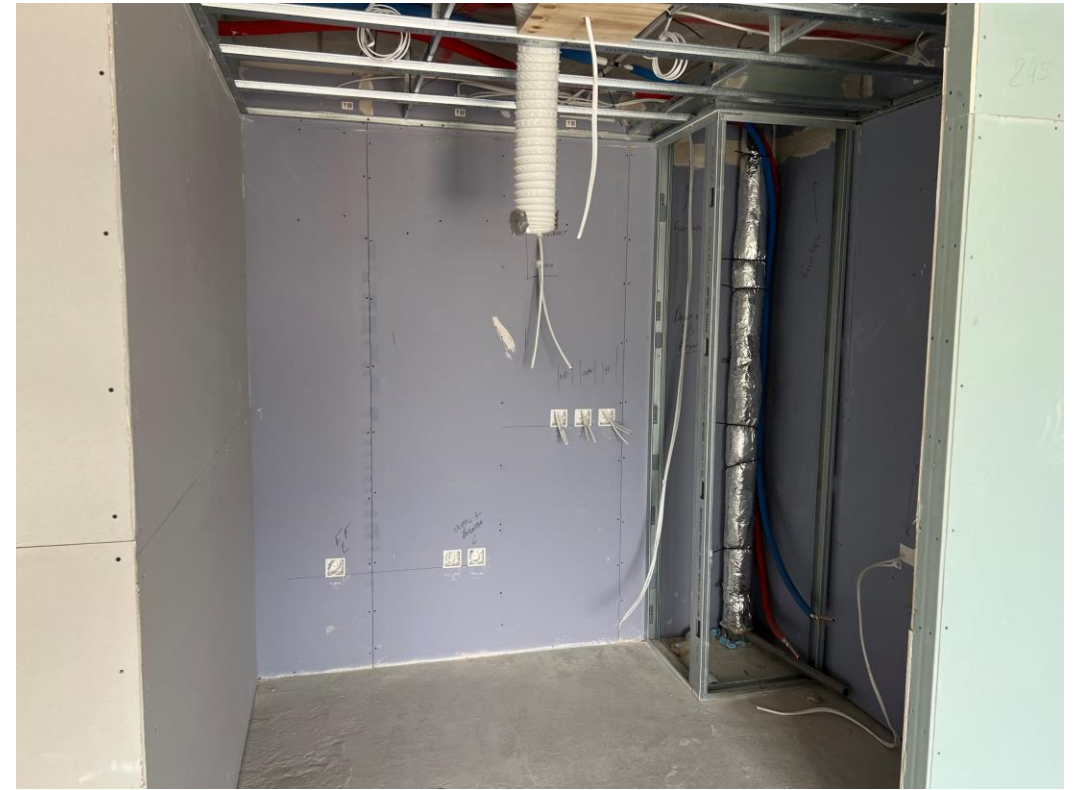
Level 3 – walls insulated and boarded
