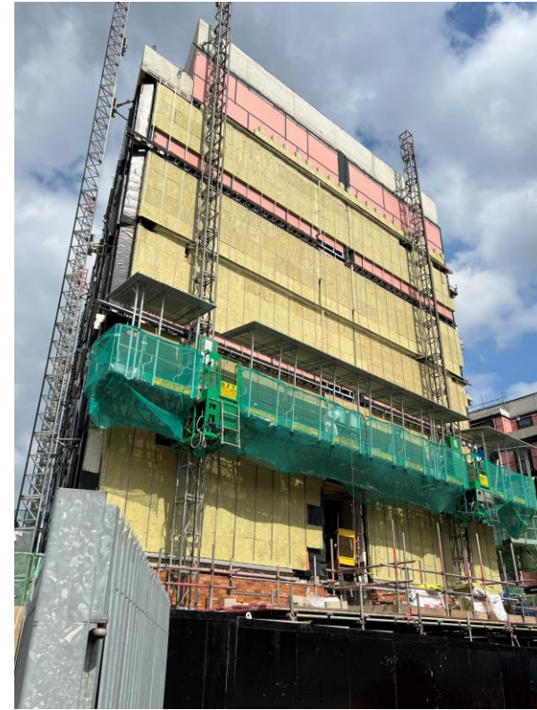
Worrall Street site view
