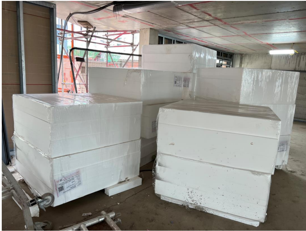
Block A roof insulation stored
