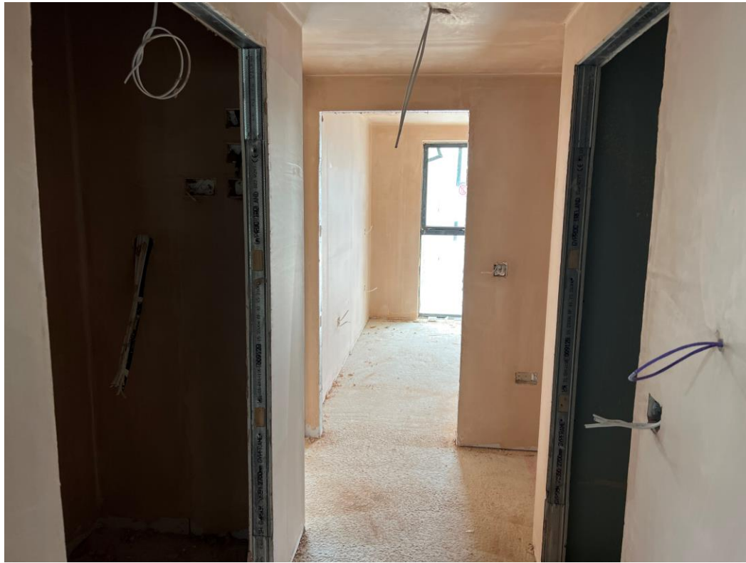
Level 1 – walls and ceilings plastered
