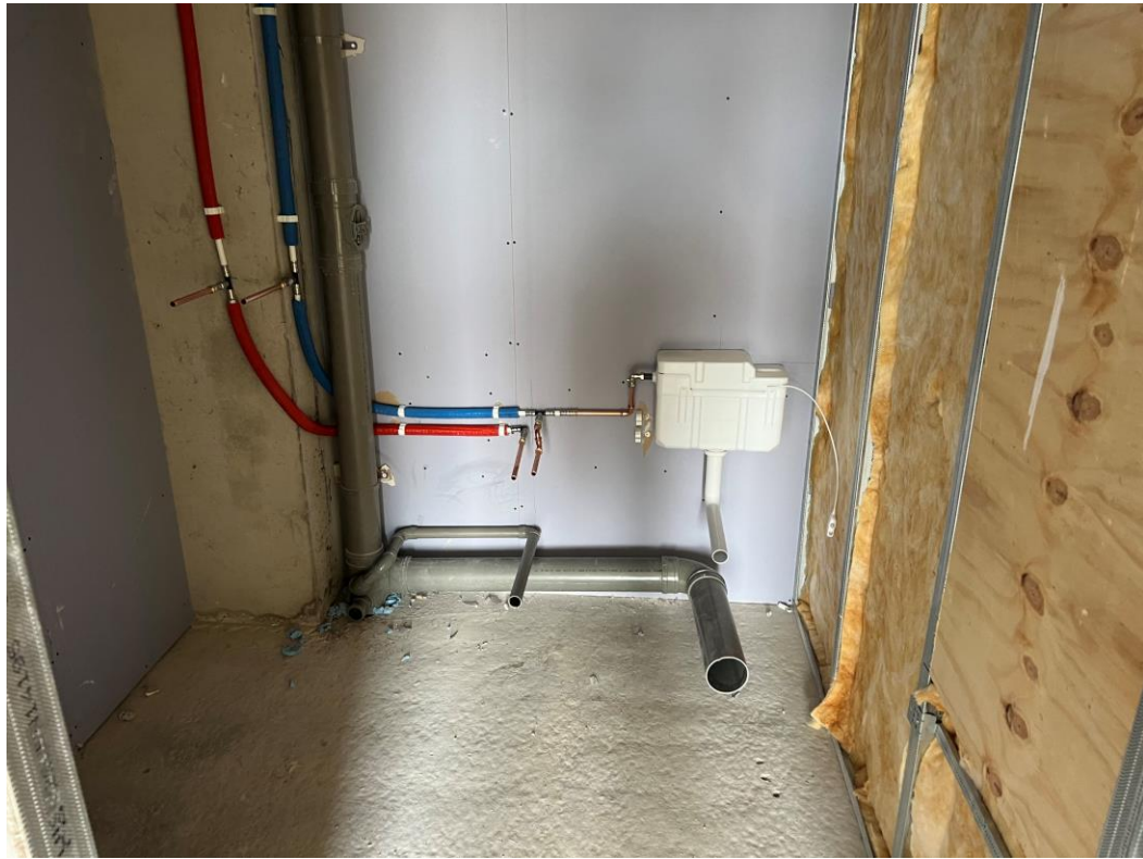
Level 5 – 1 st fix plumbing
