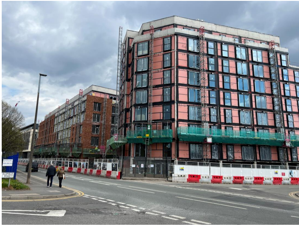
Ordsall Lane site view
