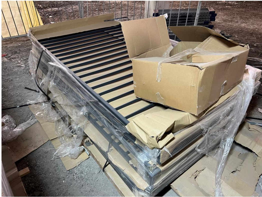
Block B Juliette balcony railings stored
