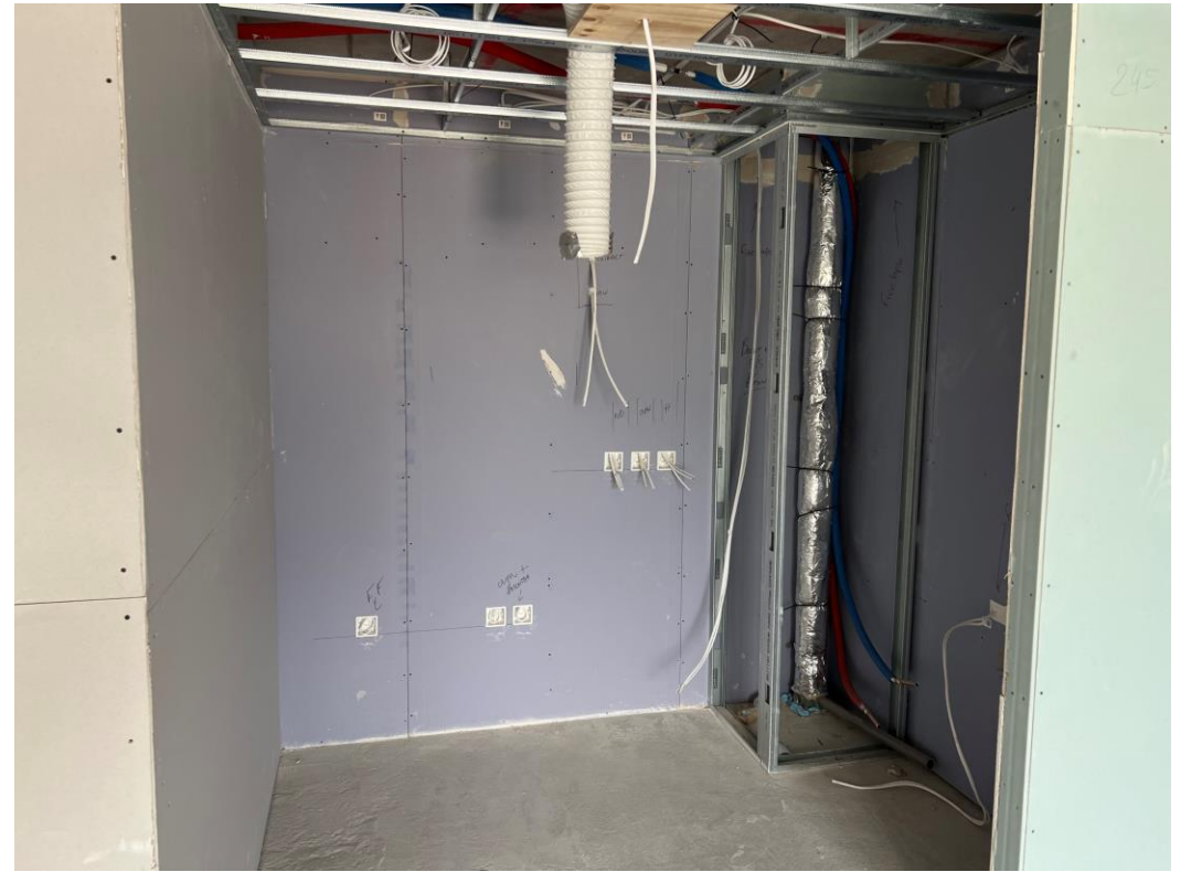
Level 3 – walls insulated and boarded
