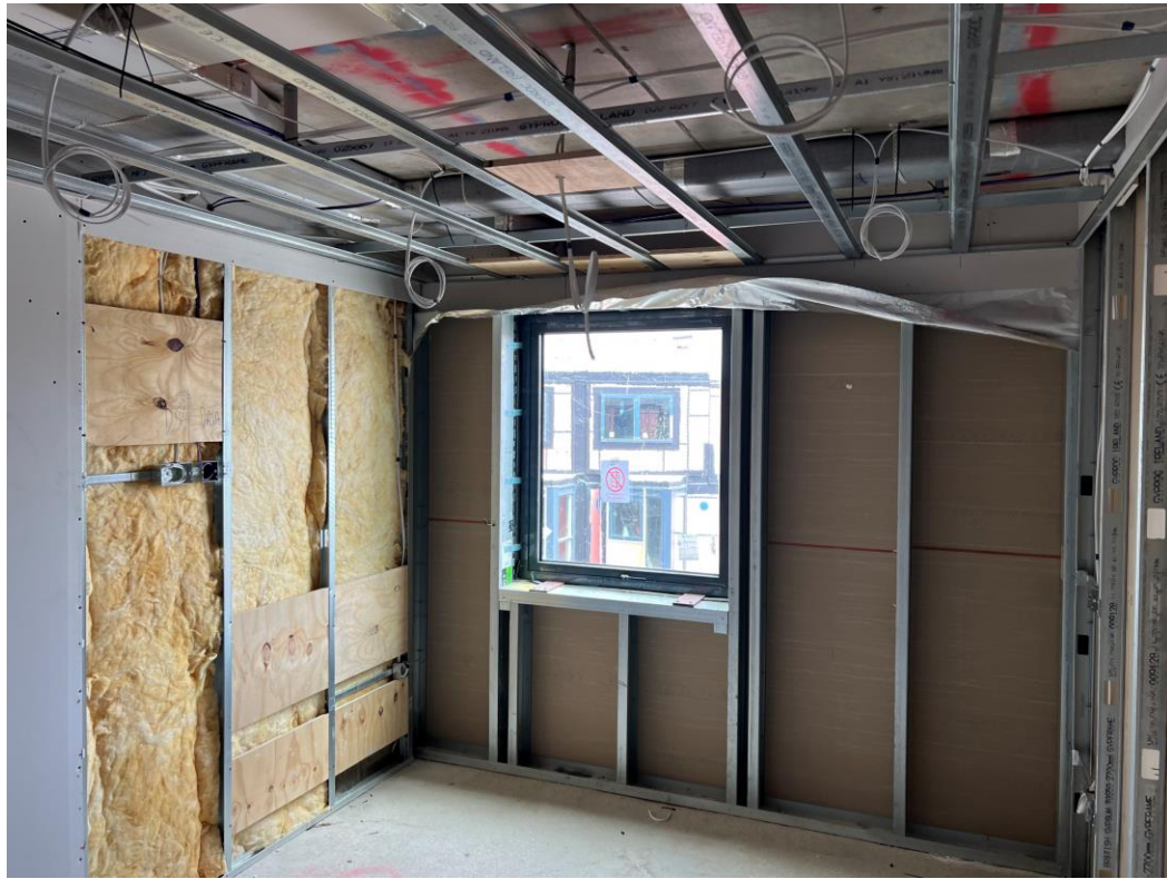
Level 6 – corridor and apartment walls formed
