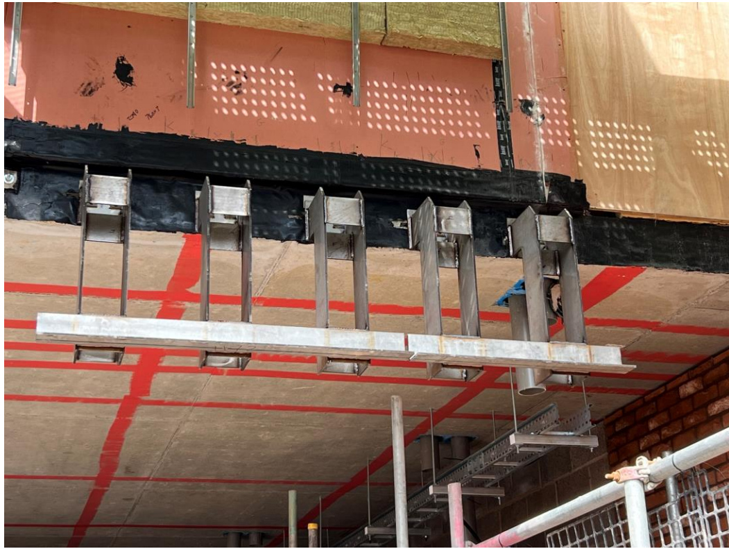
Block B masonry support
