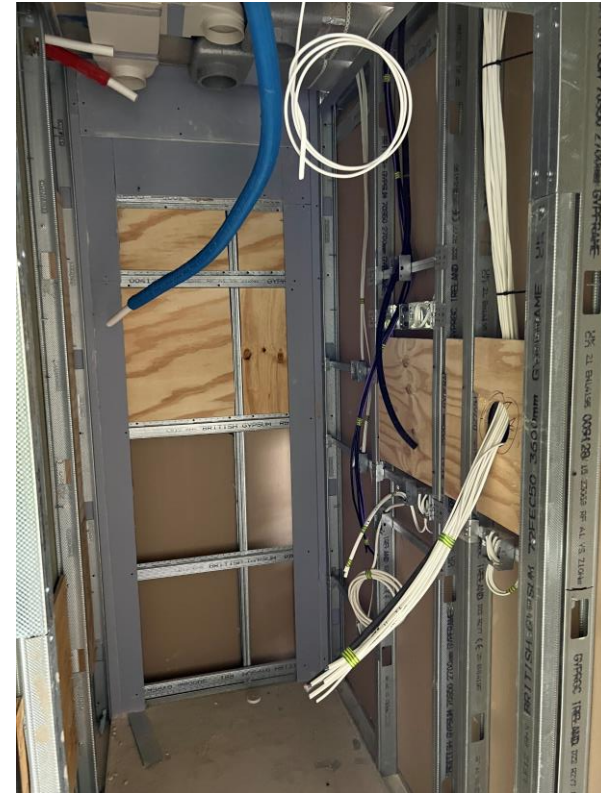
Level 5 – 1 st fix electrical
