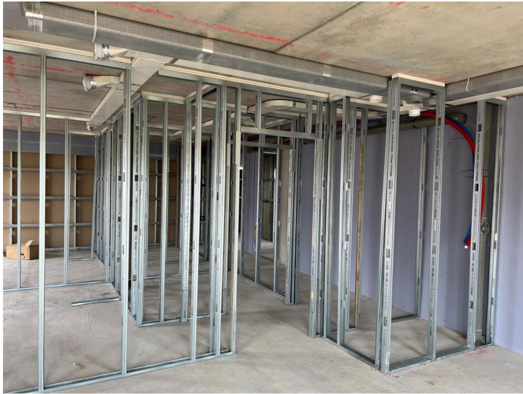
Level 7 – Apartment wall framework
