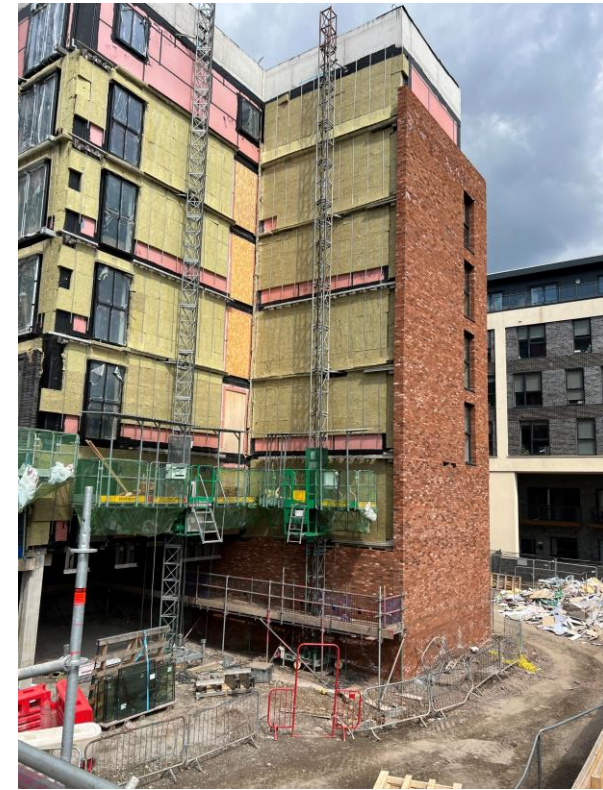
Block B wall insulation & brickwork
