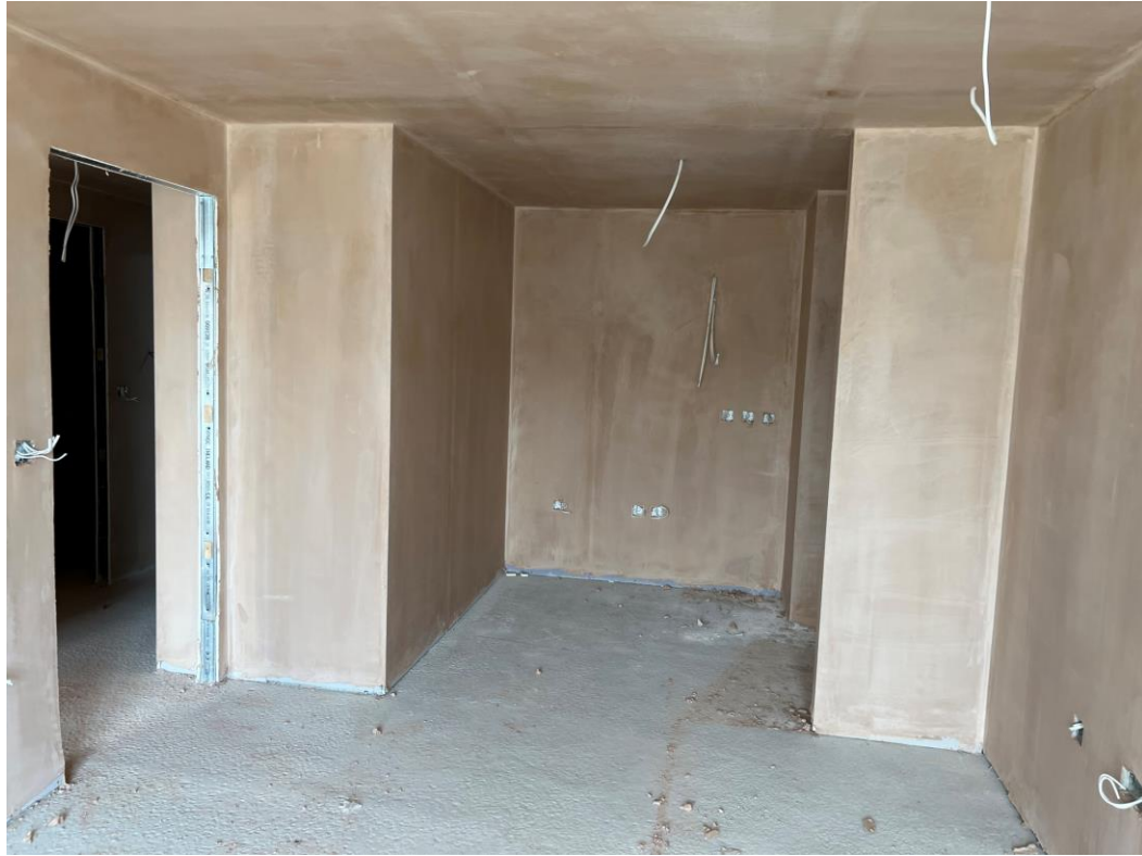
Level 1 – walls and ceilings plastered
