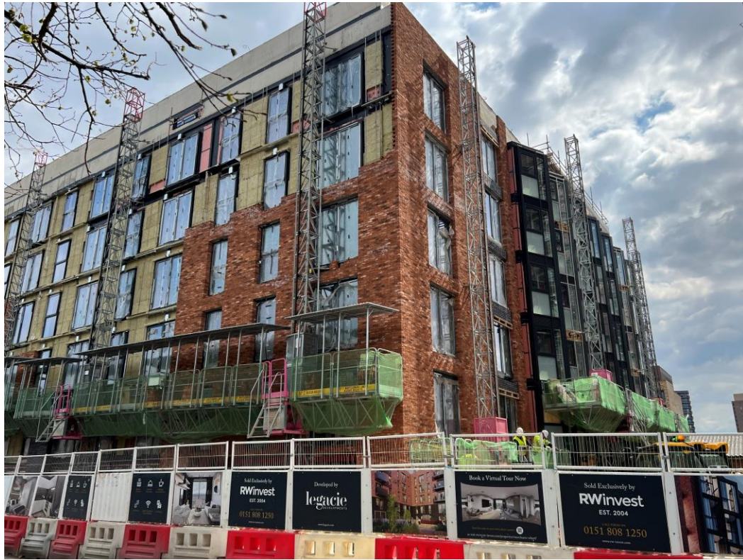
Ordsall Lane site view
