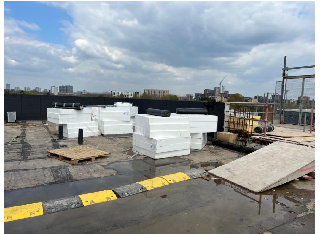
Block B main roof covering preparation
