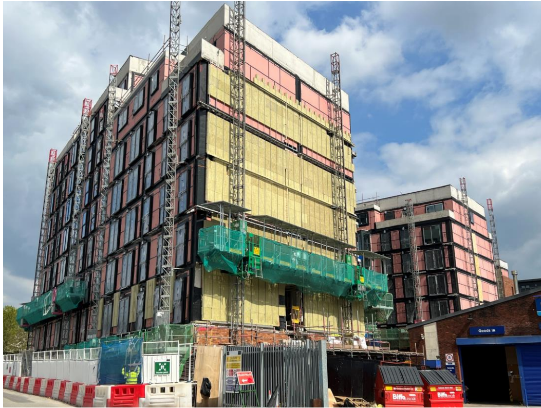
Worrall Street site view
