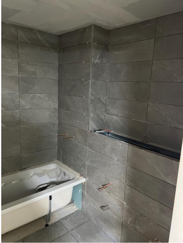
Wall and floor tiling ongoing
