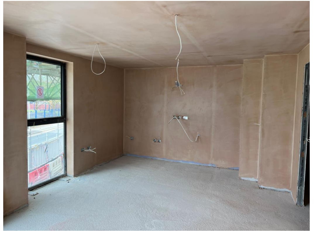
Level 1 – walls and ceilings plastered
