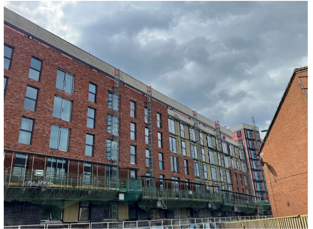
Ordsall Lane site view
