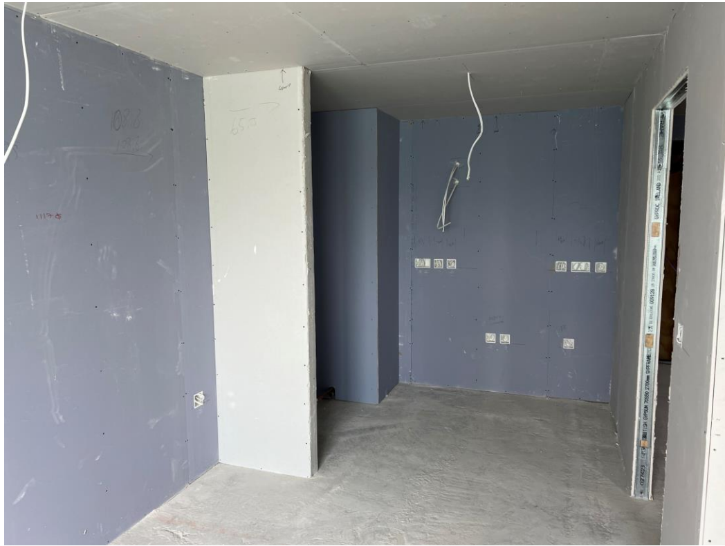
Level 2 – ceilings boarded
