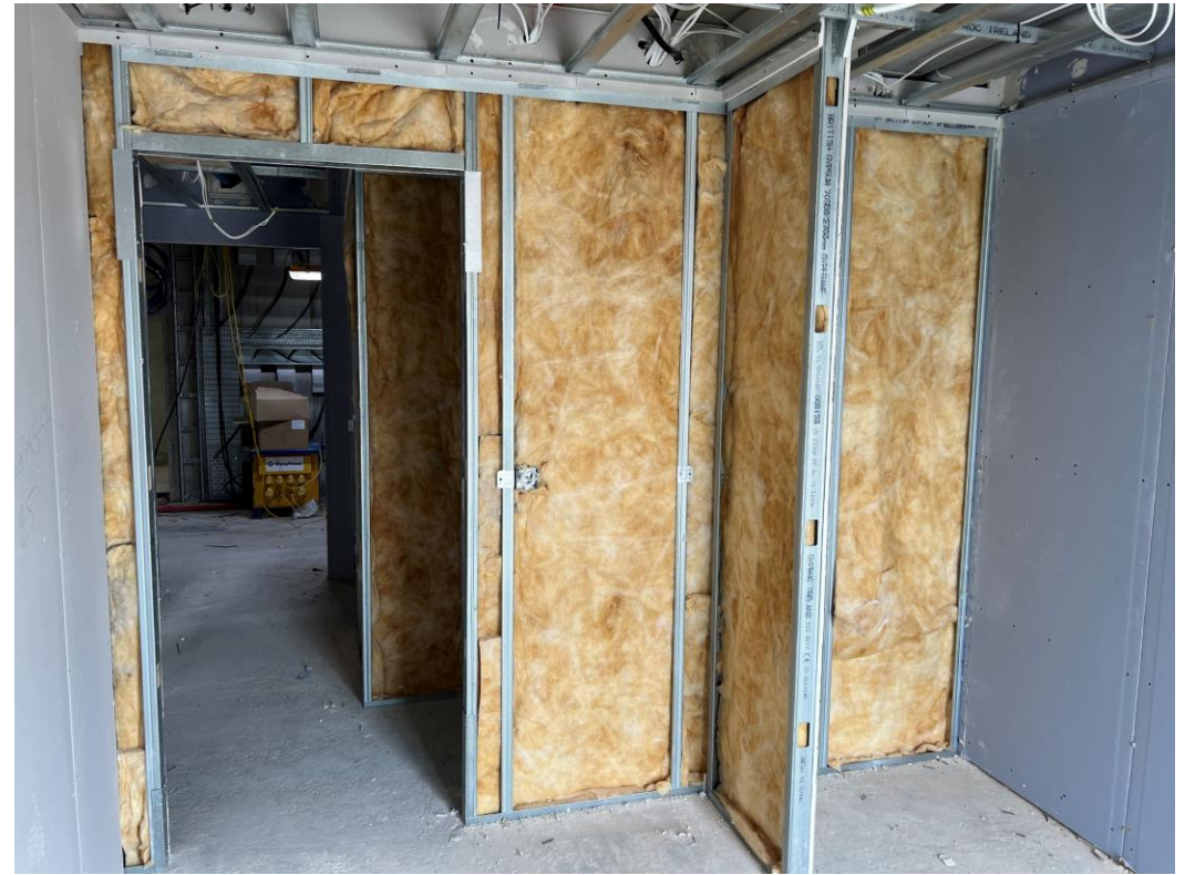
Level 4 – walls insulated ready for boarding
