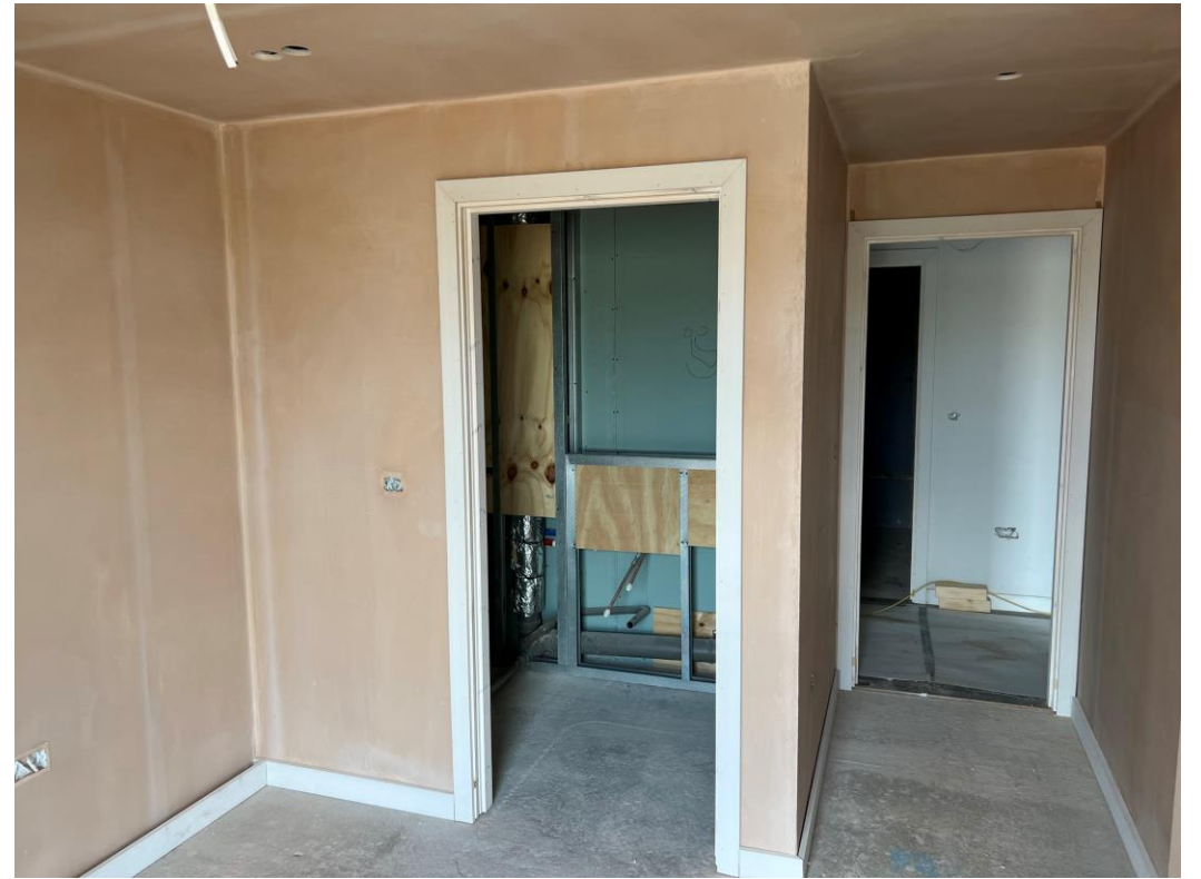
Doorframes, skirting and architrave
