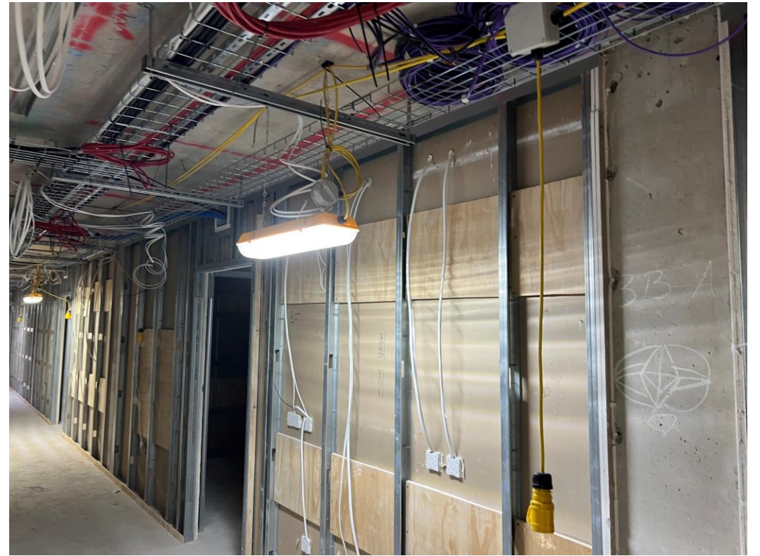
Upper floor level corridors formed
