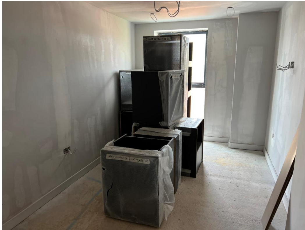
Kitchen units commenced
