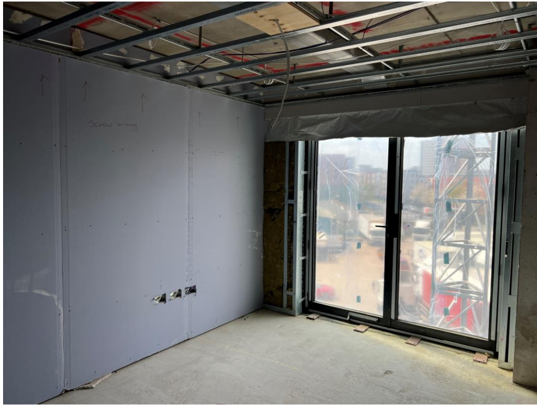
Level 3 – walls insulated and boarded
