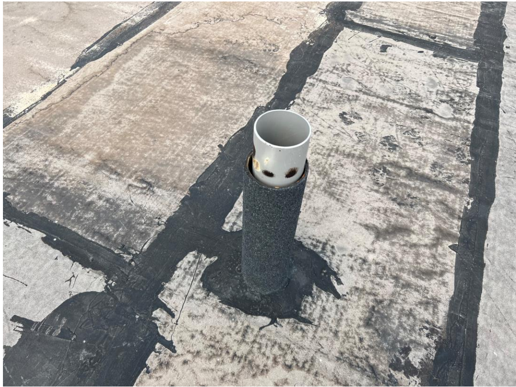
Block B main roof covering preparation
