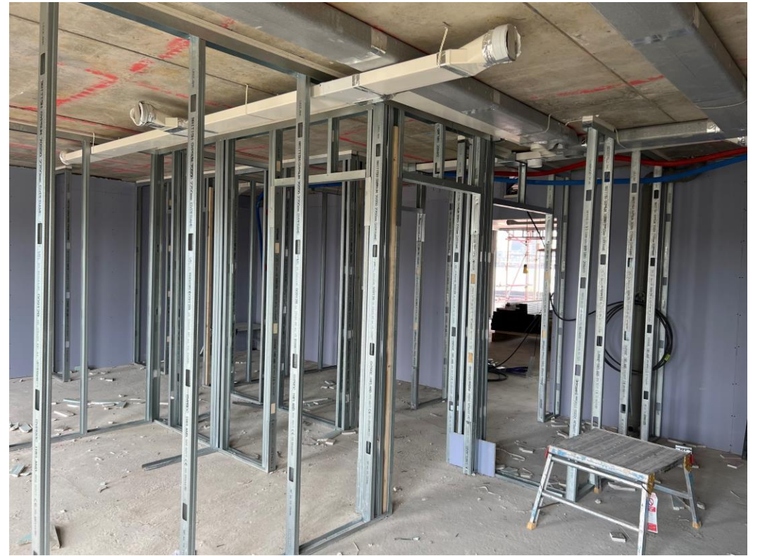
Level 7 – Apartment wall framework
