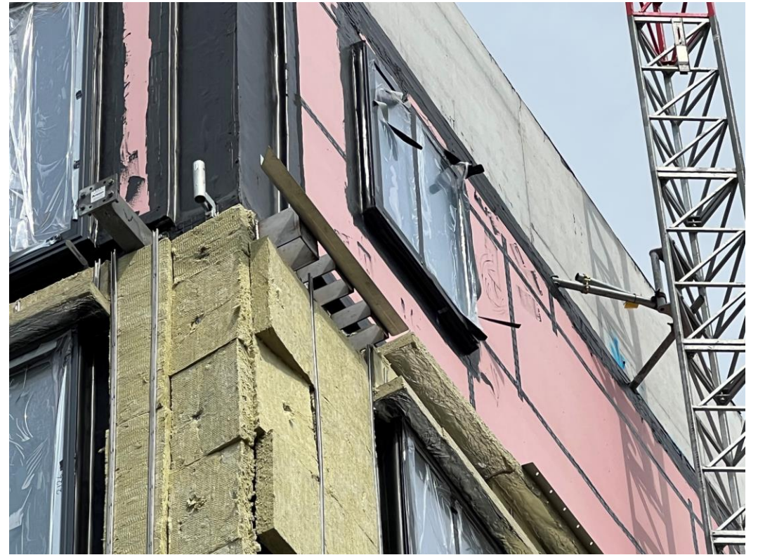
Block B masonry support
