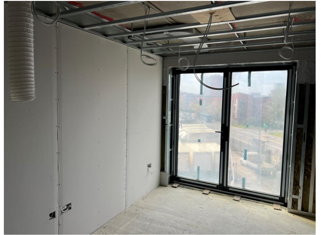
Level 3 – walls insulated and boarded
