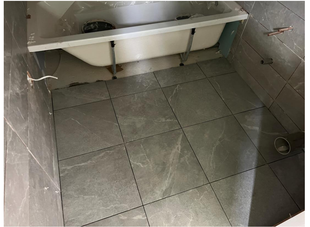
Wall and floor tiling ongoing
