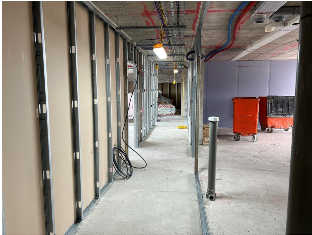
Level 8 – Corridor partitions formed
