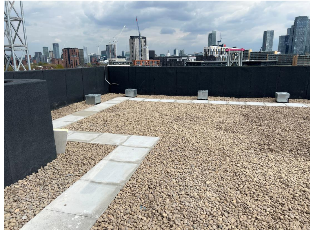
Block B inverted main roof covering preparation
