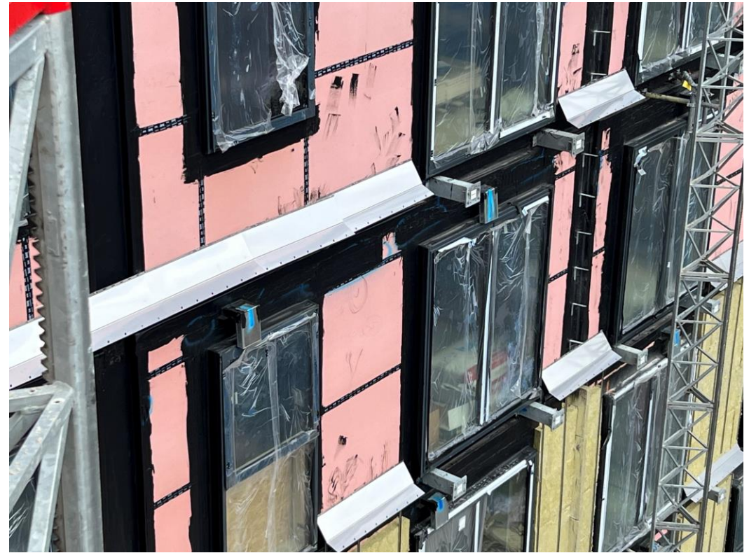
Block B cavity trays
