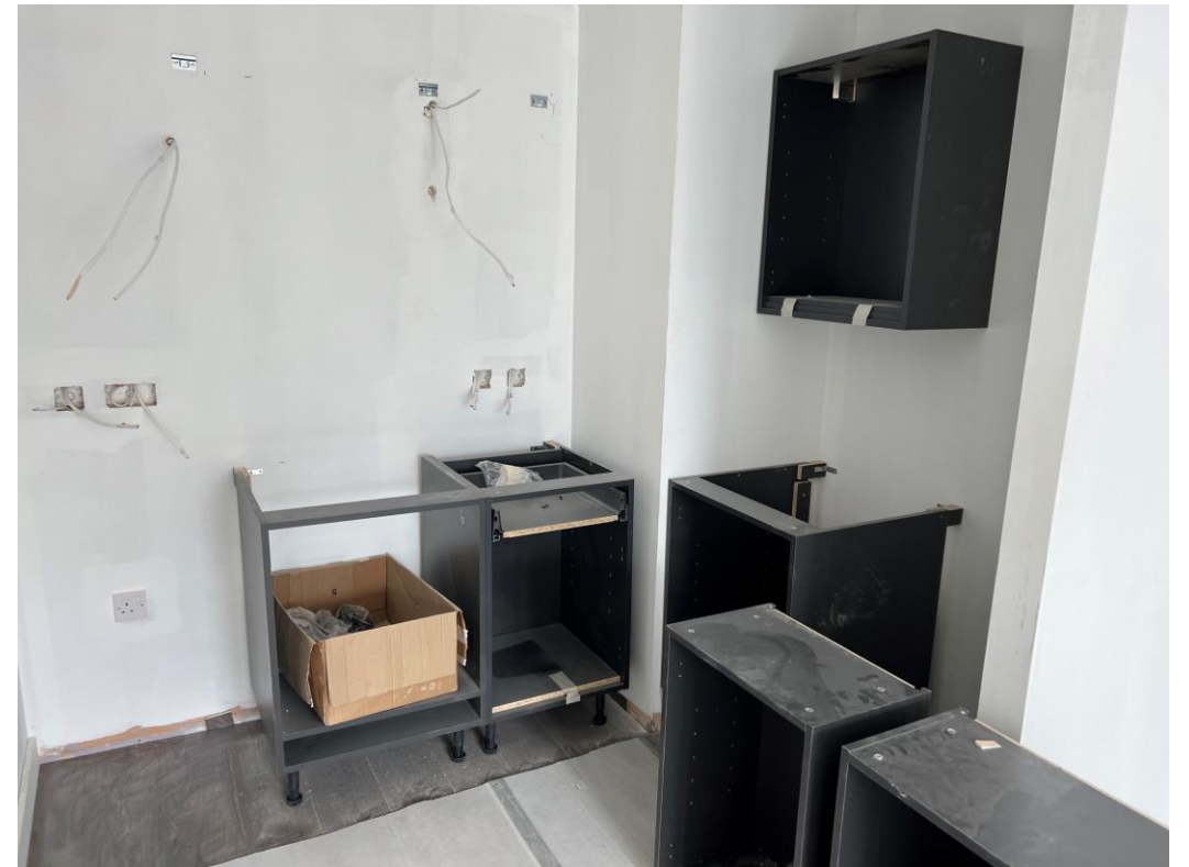
Kitchen units commenced
