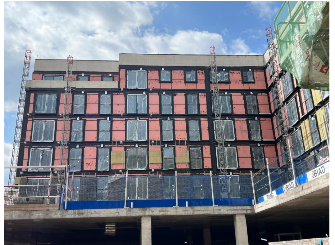
Block B wall insulation & brickwork
