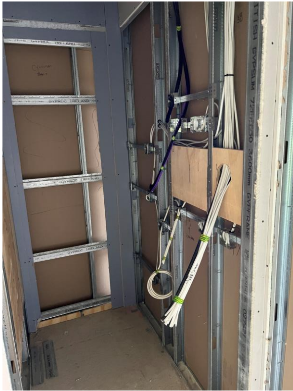
Level 6 – 1 st fix electrical
