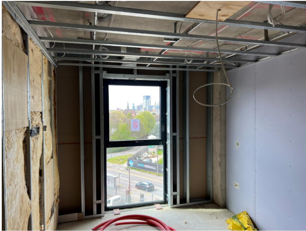
Level 5 – ceiling installation
