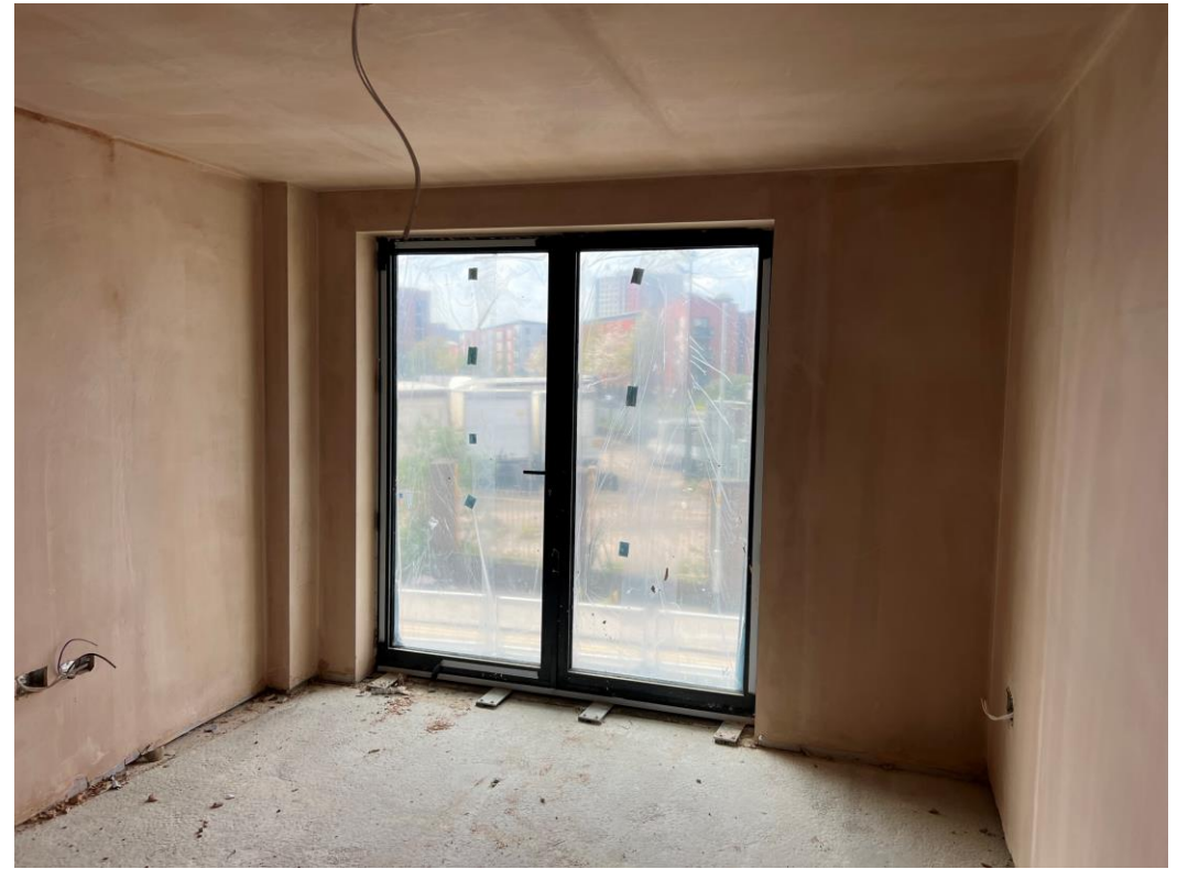
Level 1 – walls and ceilings plastered
