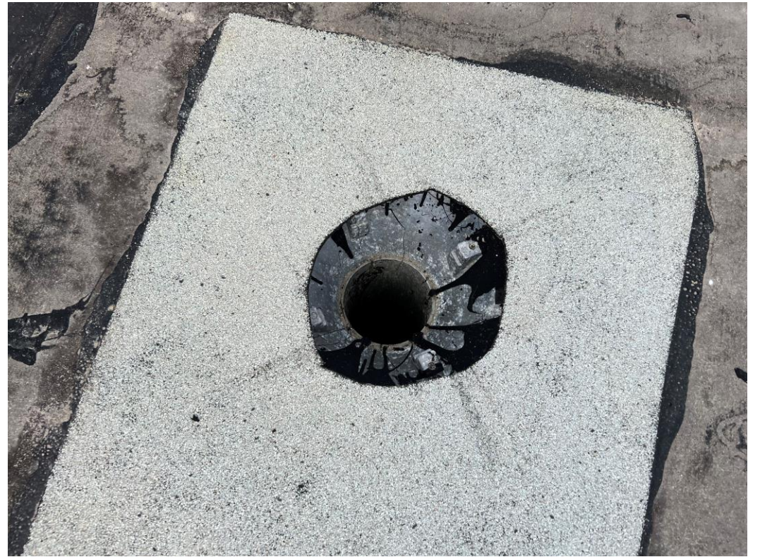
Block B main roof covering preparation
