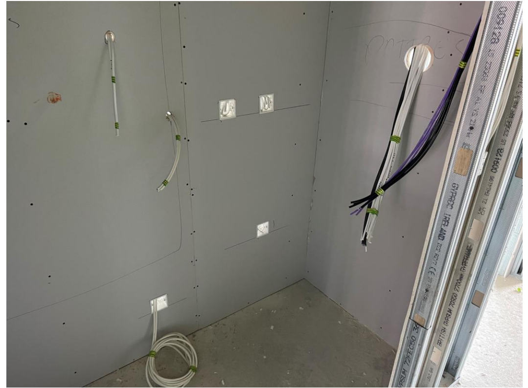
Level 6 – 1 st fix electrical
