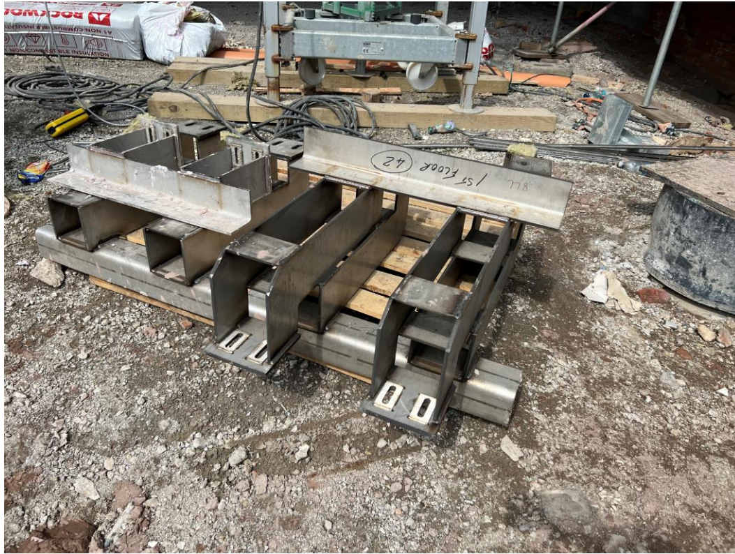
Block B masonry support
