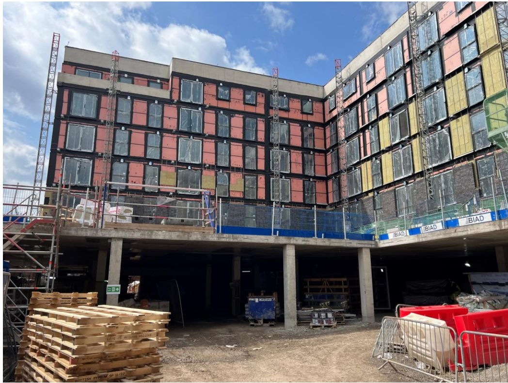
Block B wall insulation & brickwork
