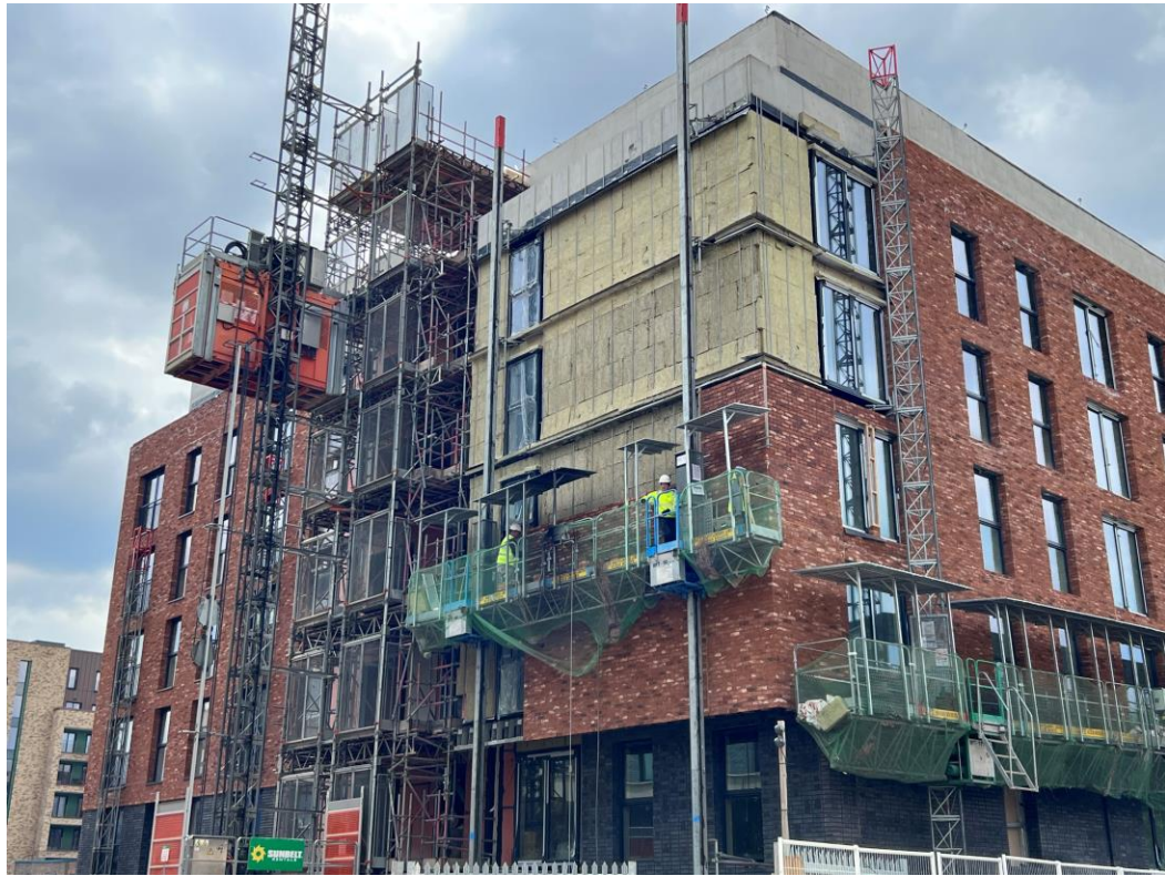
Ordsall Lane site view
