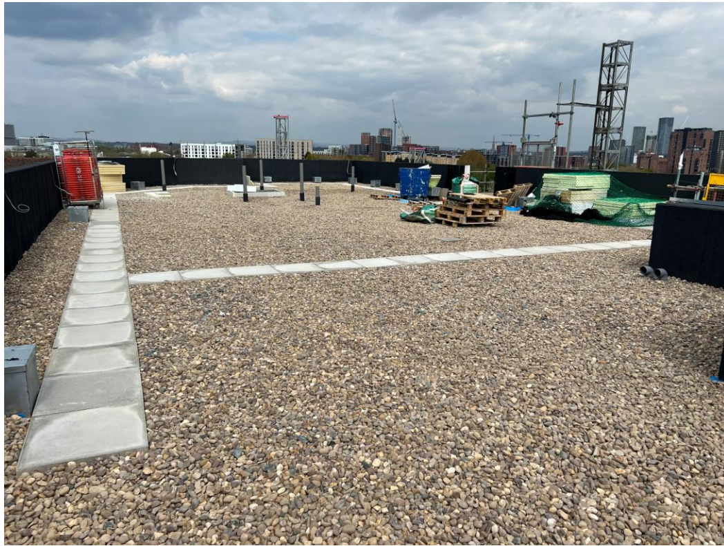
Block A inverted main roof system complete
