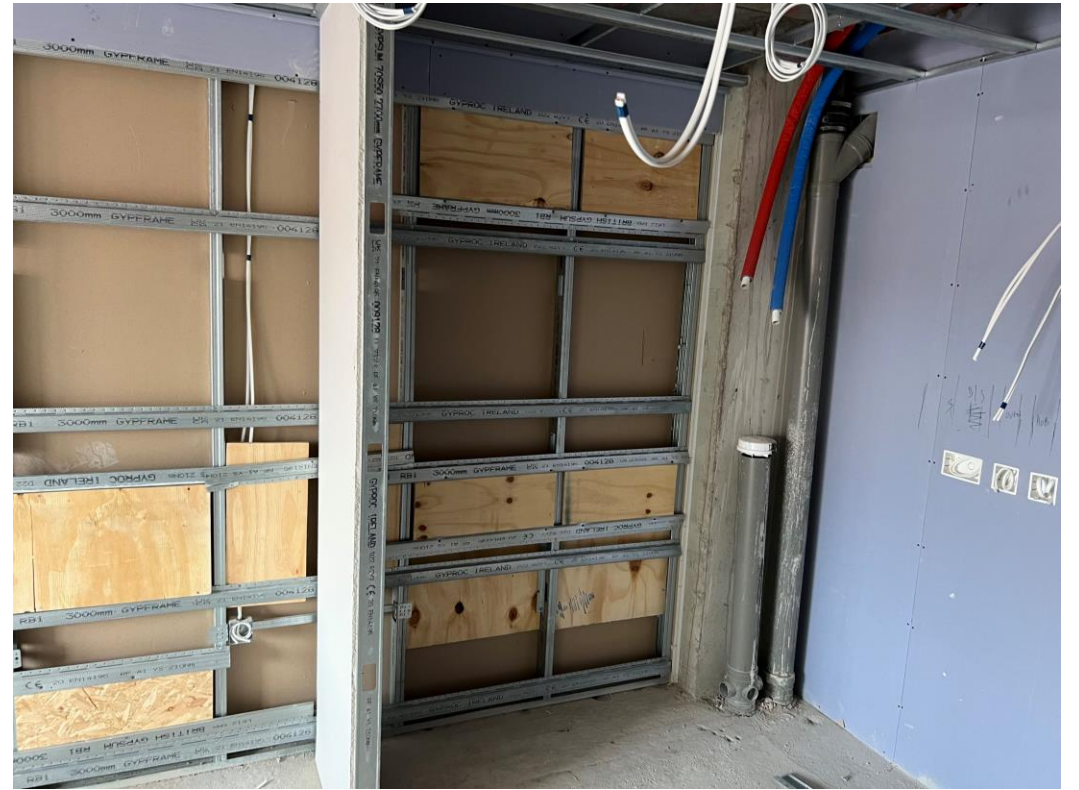
Level 6 – corridor and apartment walls formed
