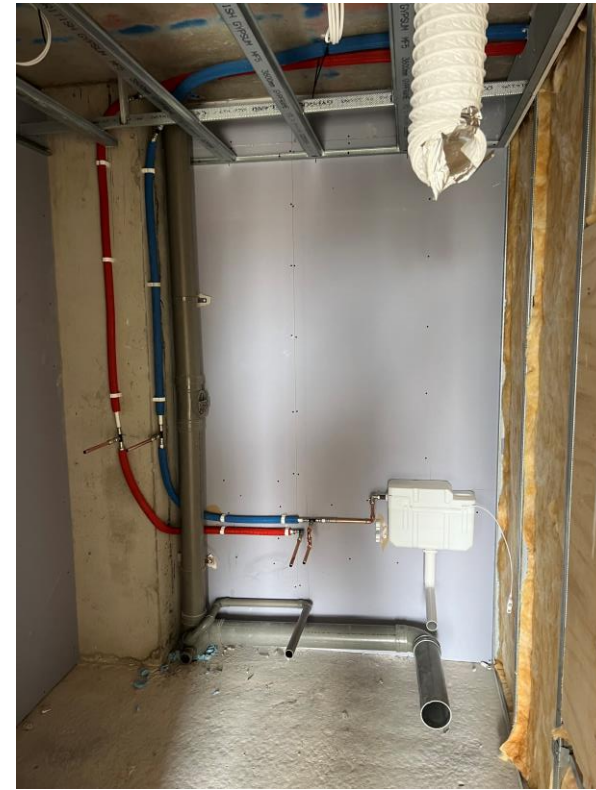
Level 5 – 1 st fix plumbing
