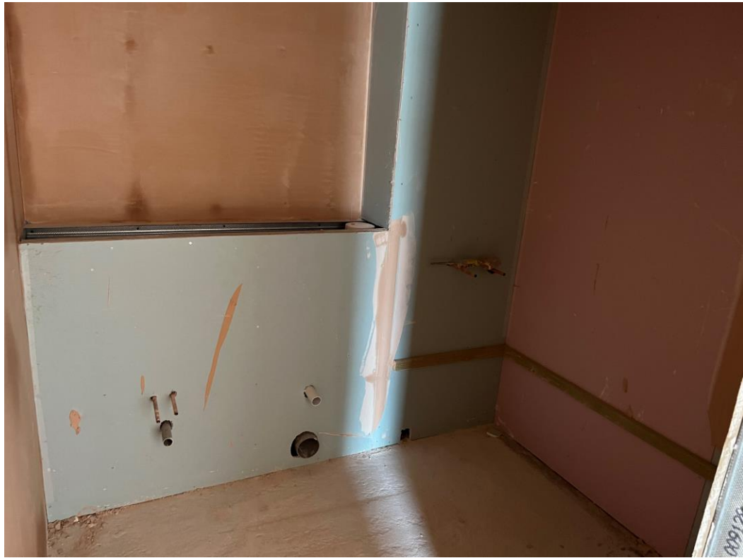
Level 1 – walls and ceilings plastered
