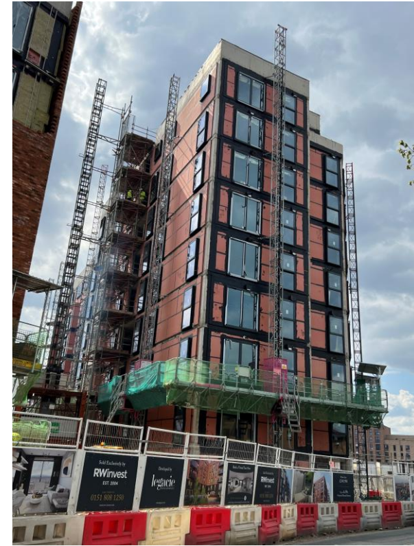
Ordsall Lane site view
