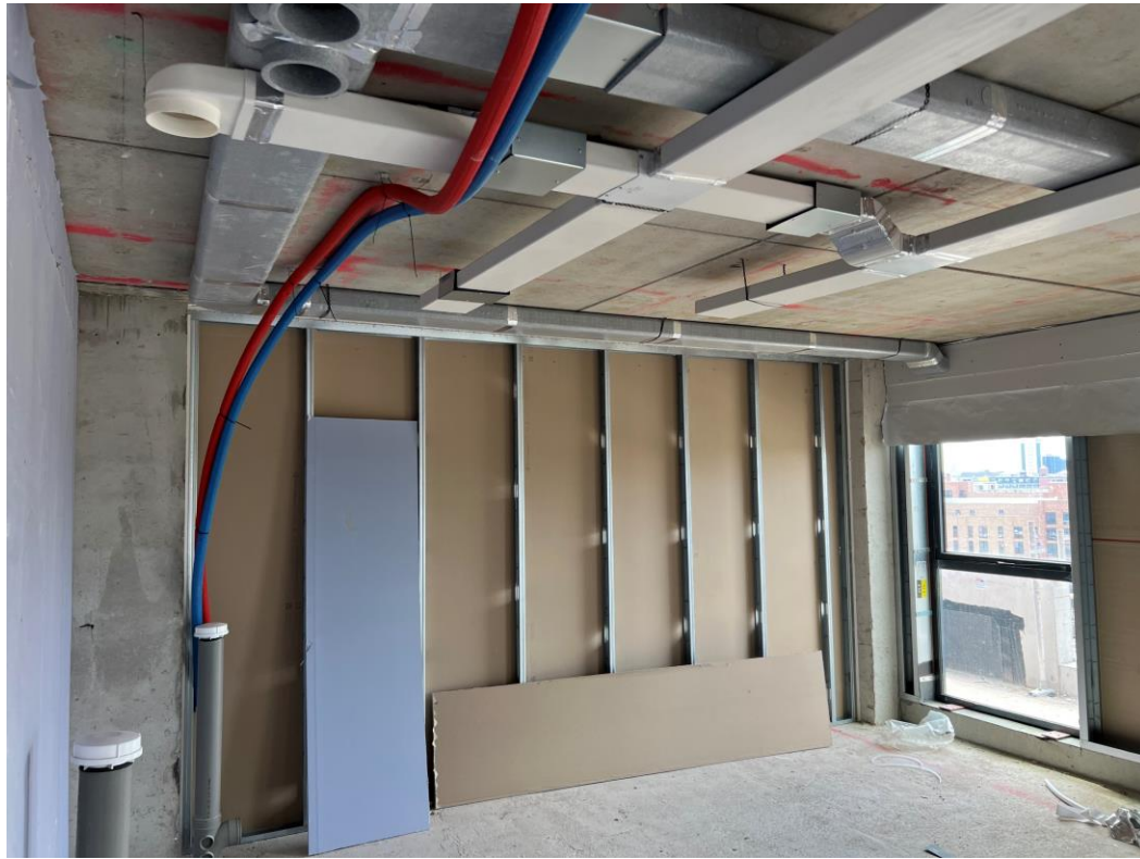
Level 8 – Corridor partitions formed
