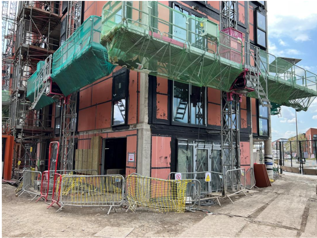
Block A weatherboarding & windows installed
