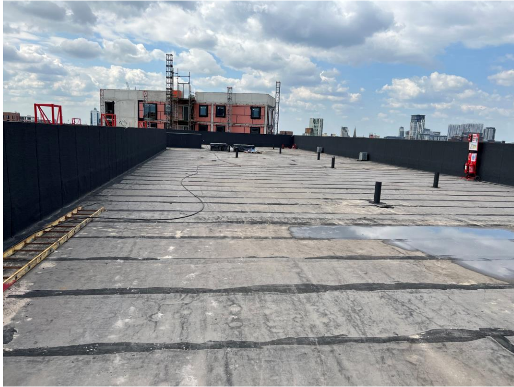
Block B main roof covering preparation
