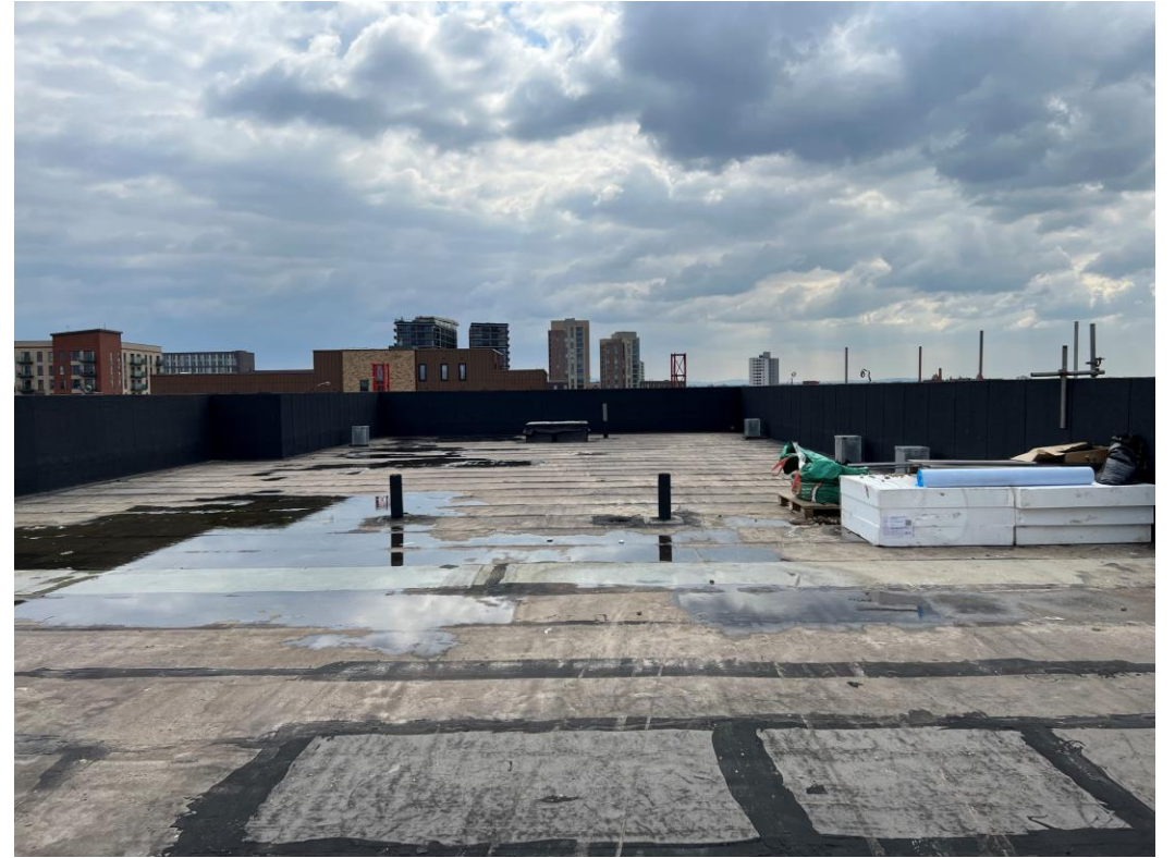
Block B main roof covering preparation
