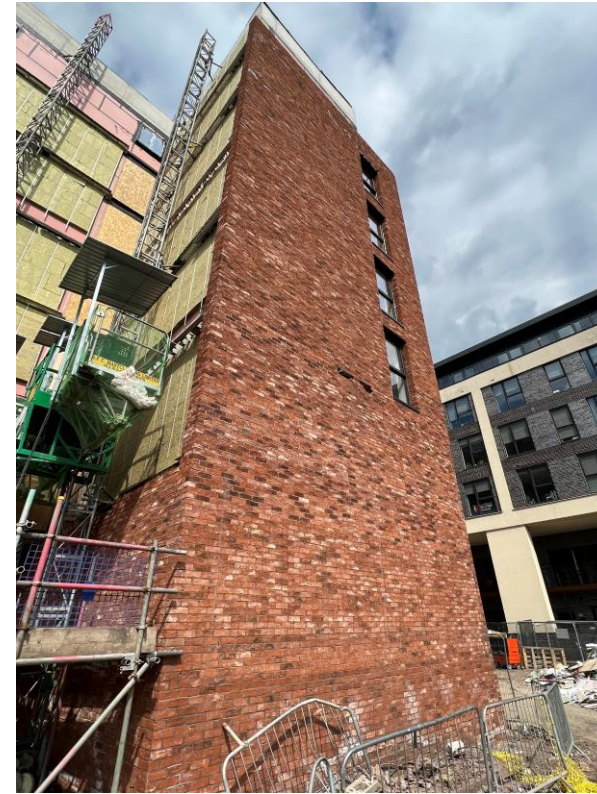
Block B masonry support
