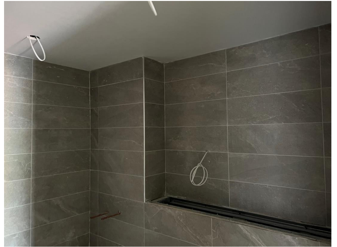
Wall and floor tiling ongoing
