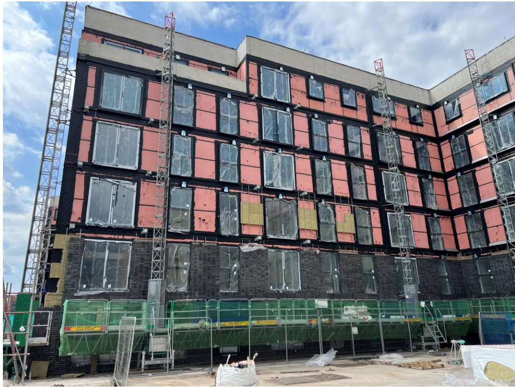
Block B wall insulation & brickwork
