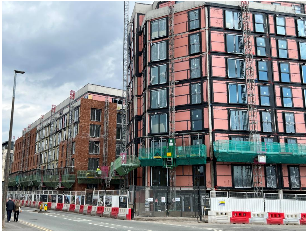
Ordsall Lane site view
