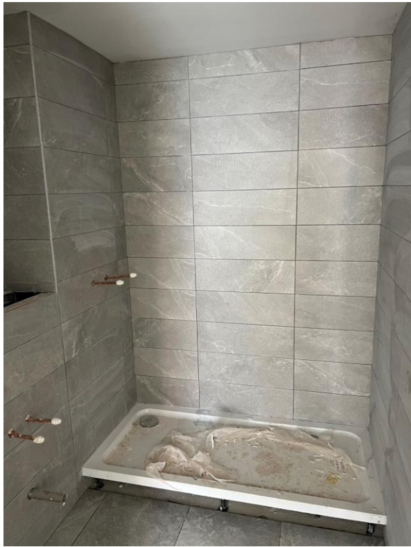
Wall and floor tiling ongoing
