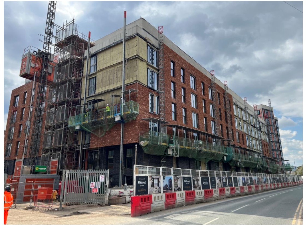
Ordsall Lane site view
