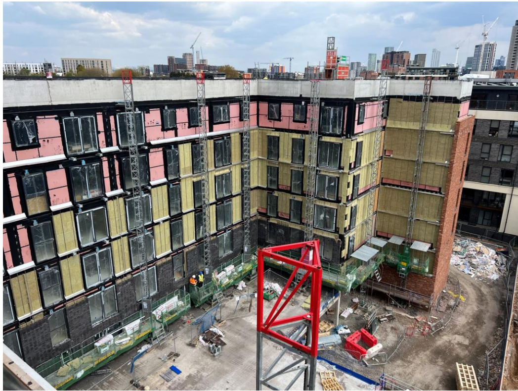
Block B wall insulation & brickwork
