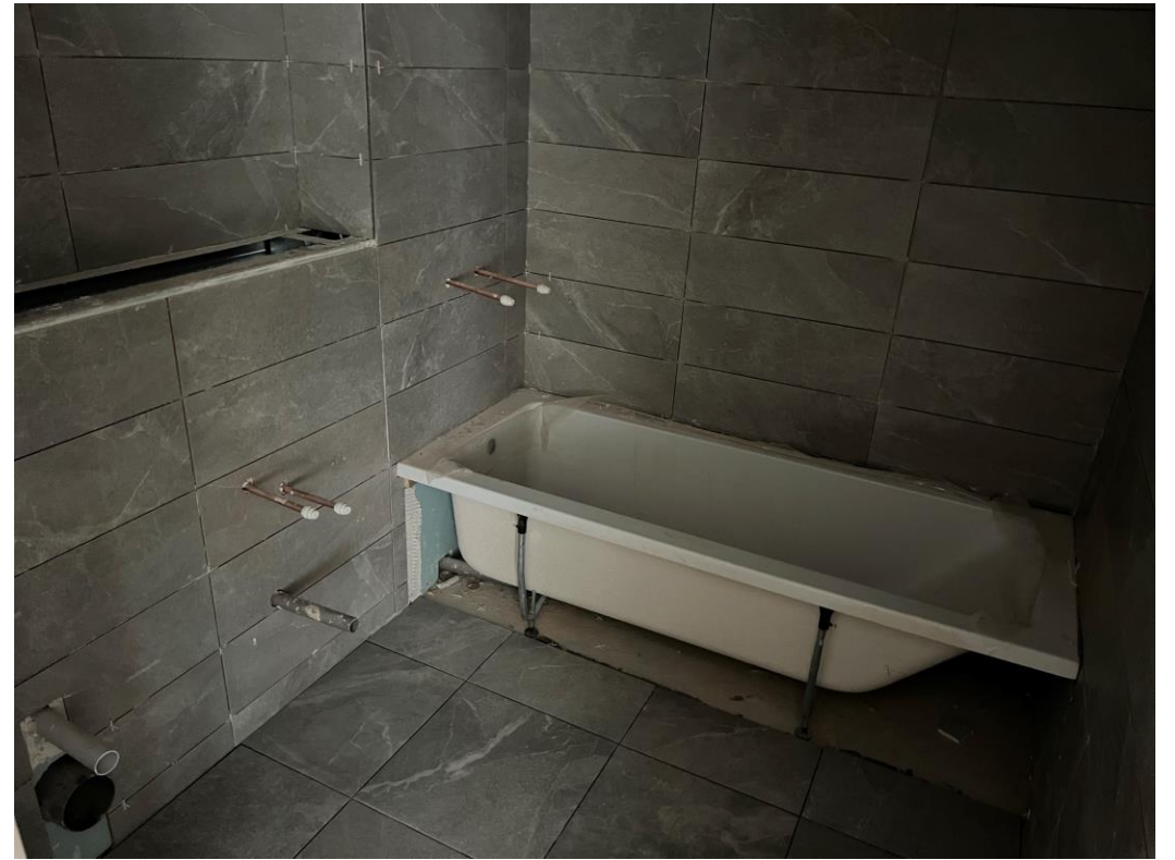
Wall and floor tiling ongoing
