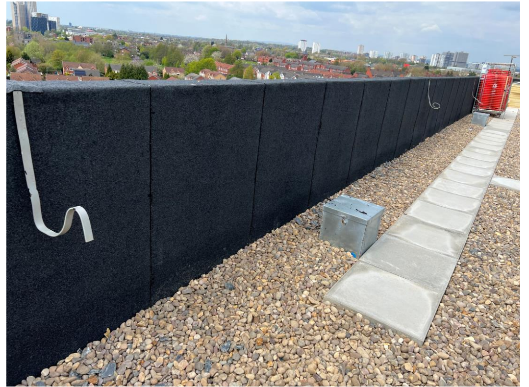
Block B inverted main roof covering preparation
