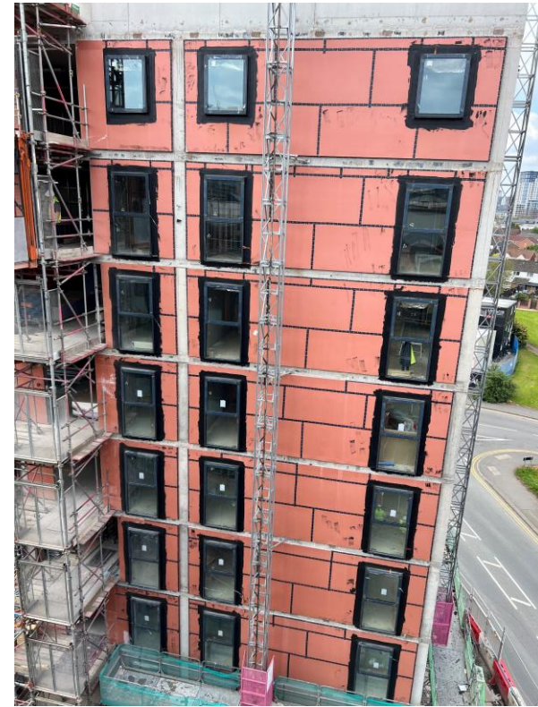
Block A weatherboarding & windows installed
