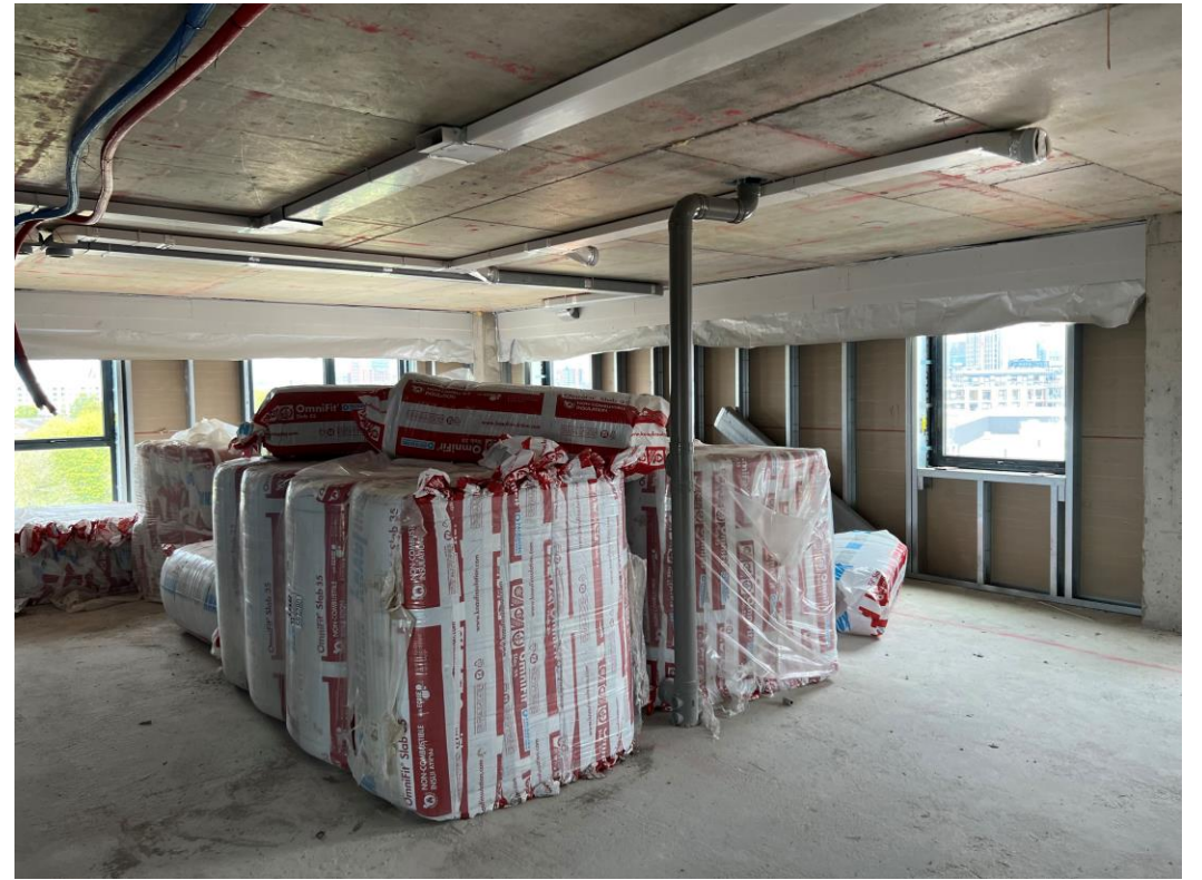
Level 8 – wall insulation
