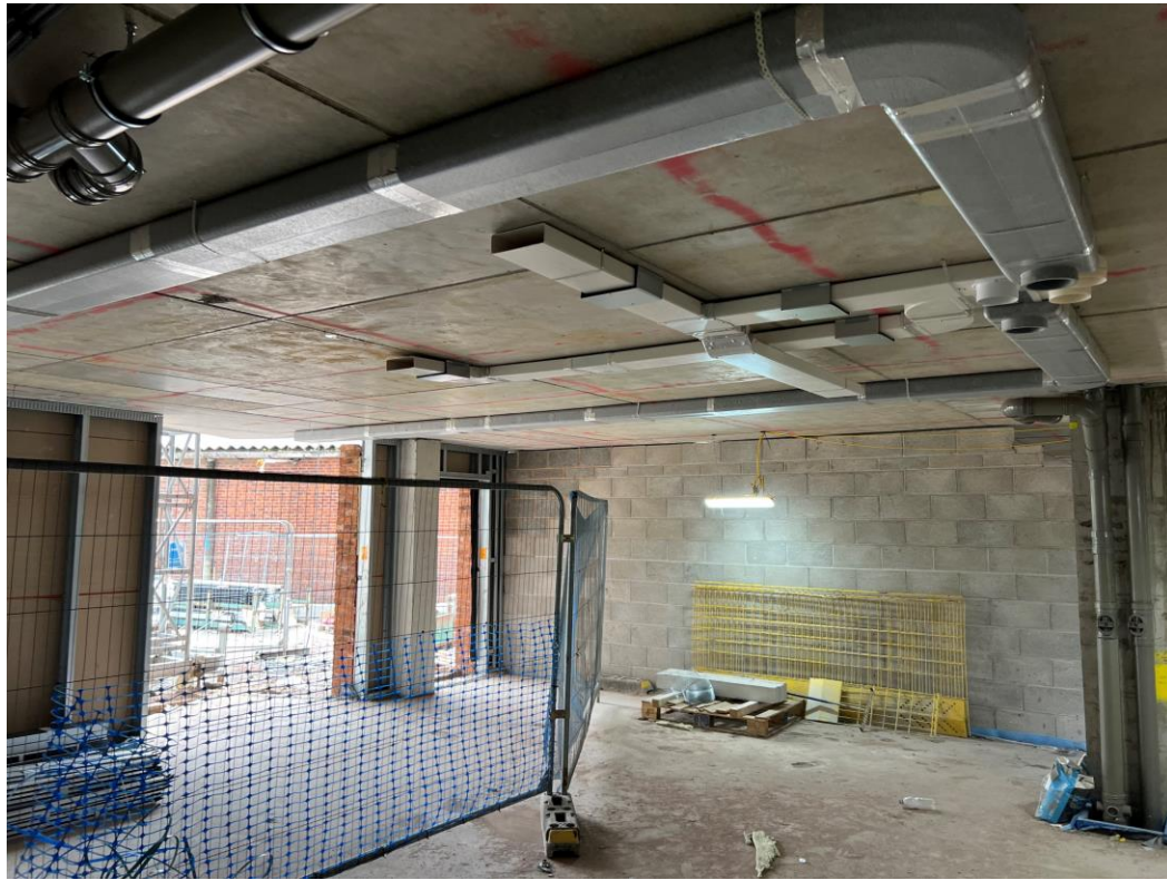
Ground floor 1 st fix mechanical
