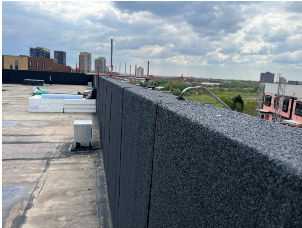
Block B main roof covering preparation
