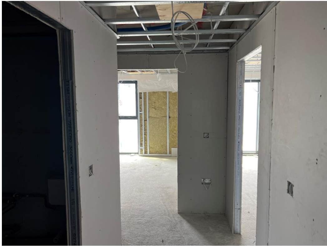
Level 3 – walls insulated and boarded
