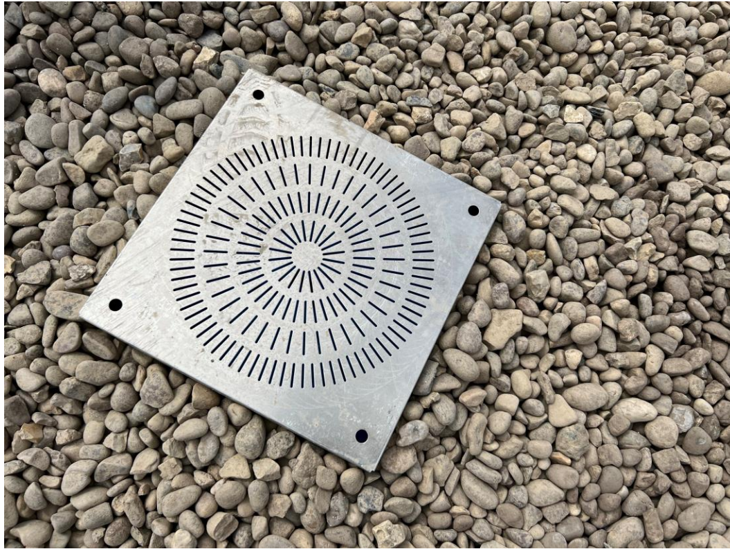
Block A inverted main roof rainwater outlet
