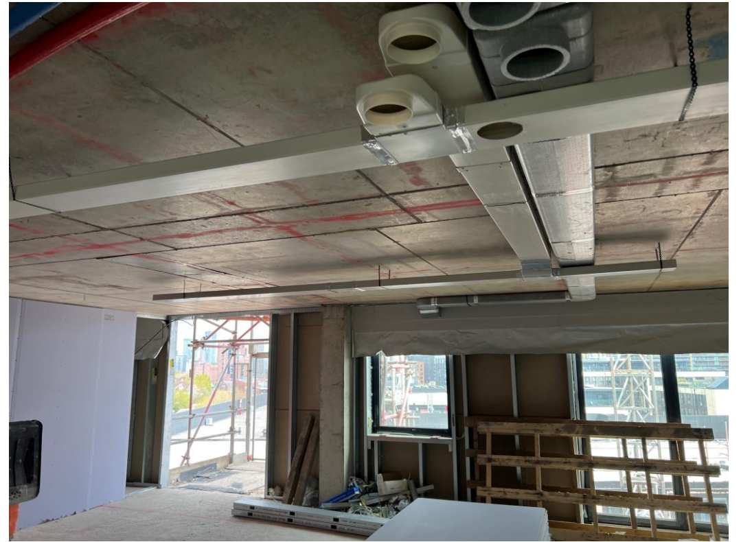
Level 8 – mechanical 1 st fix
