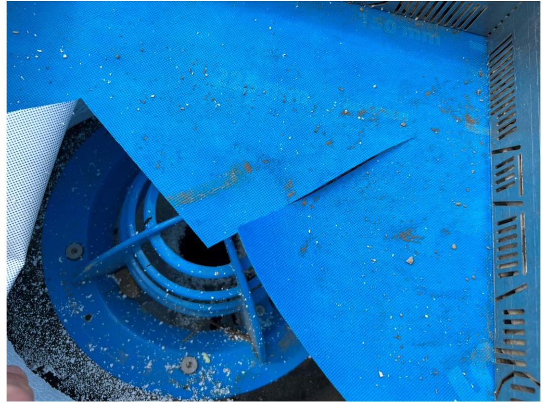
Block A inverted main roof rainwater outlet
