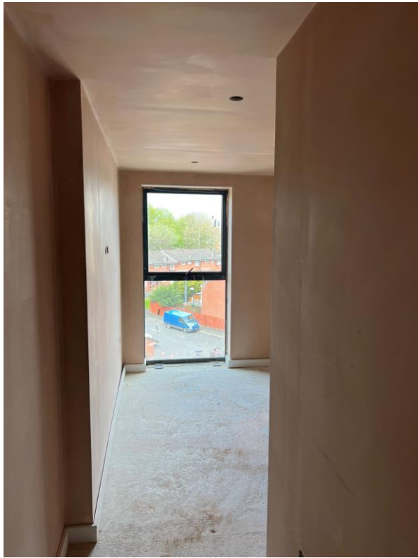
Doorframes, skirting and architrave
