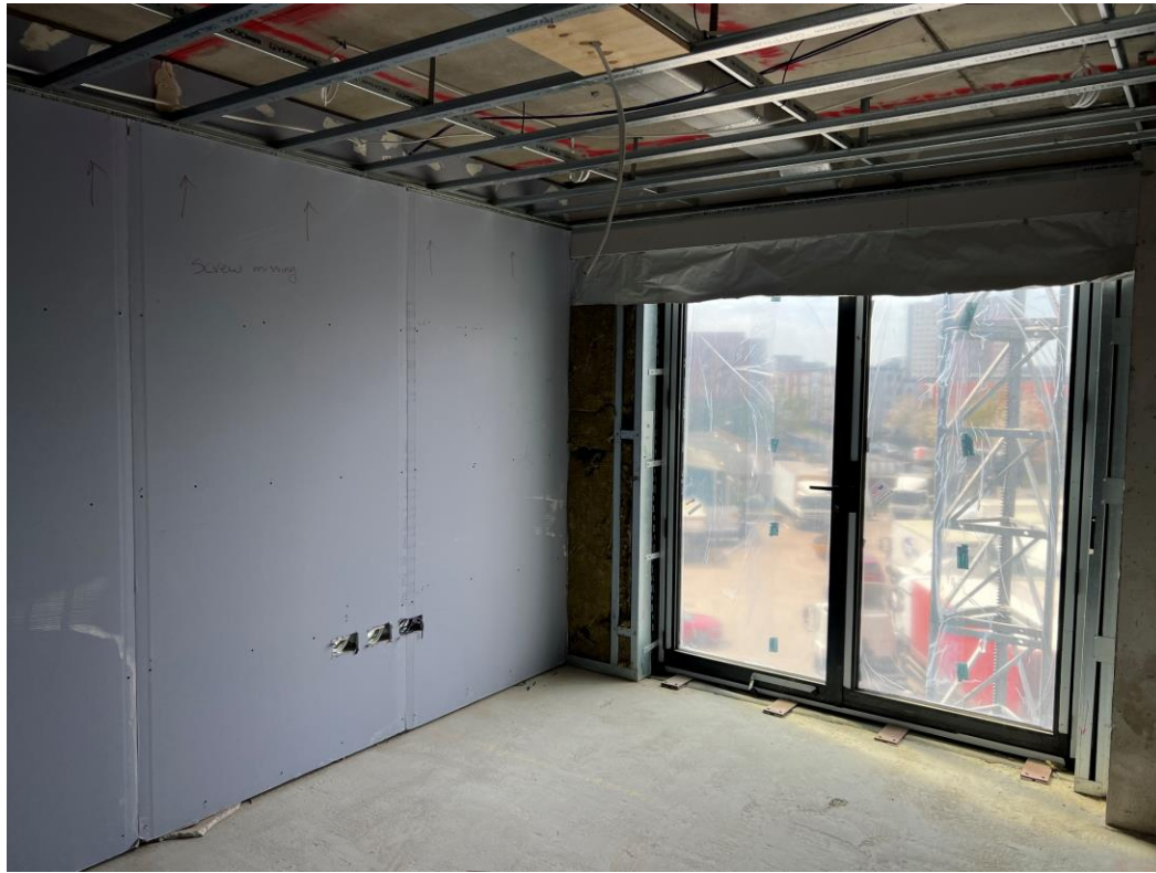
Level 3 – walls insulated and boarded
