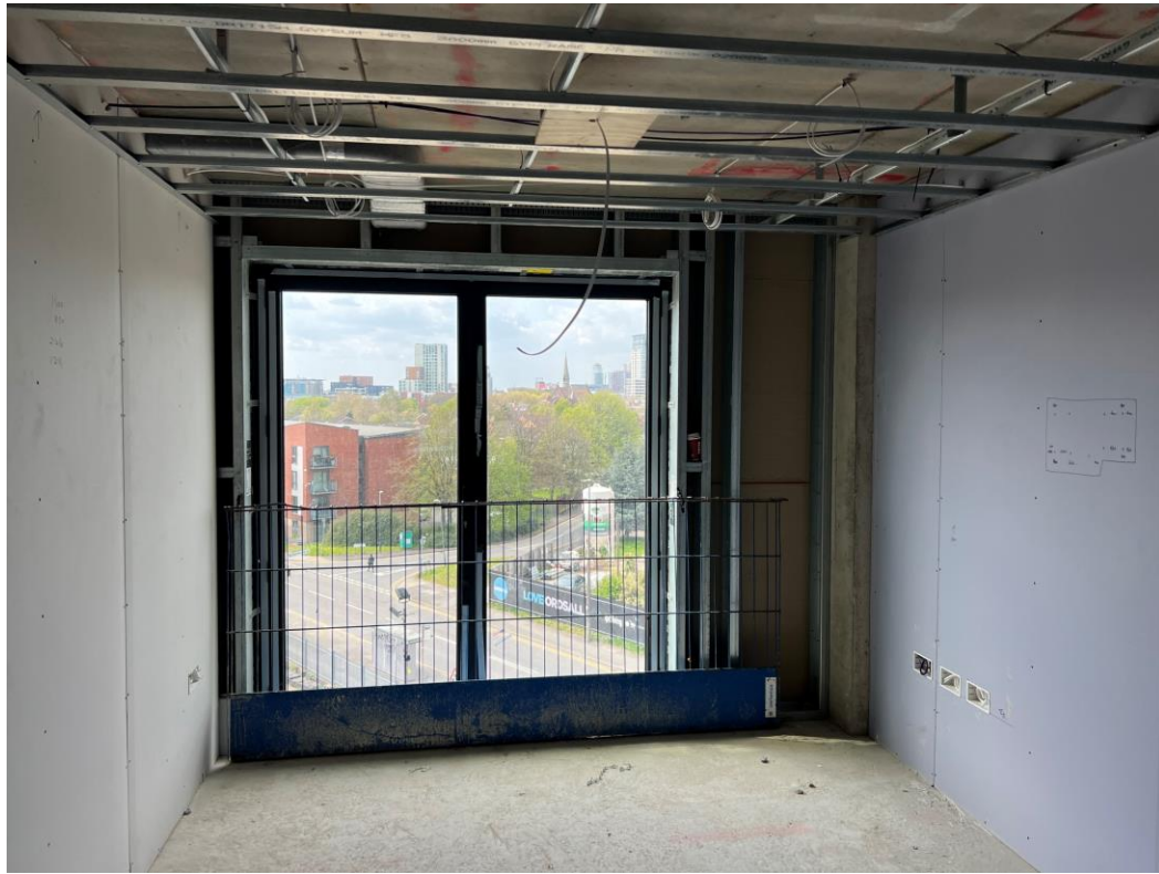
Level 5 – ceiling installation
