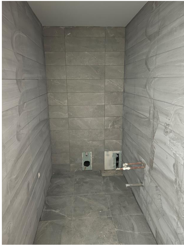
Wall and floor tiling ongoing
