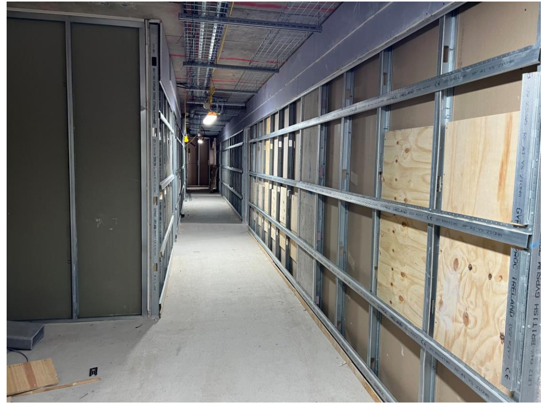
Level 6 – corridor and apartment walls formed
