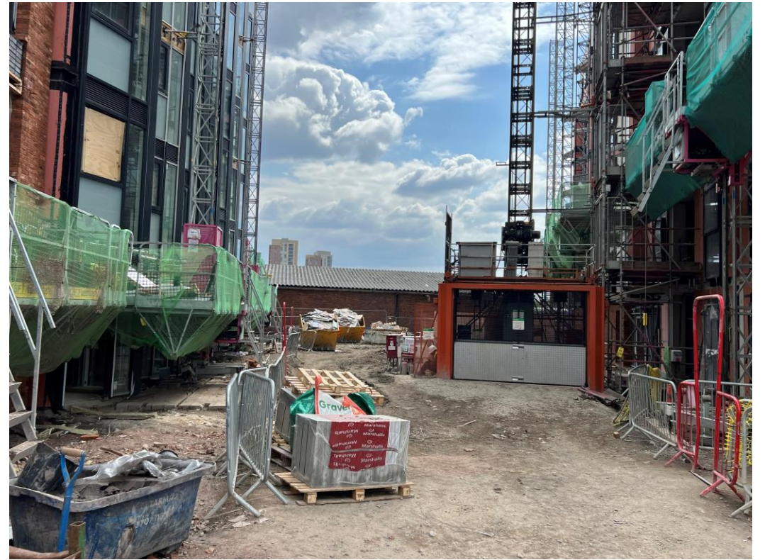
Block A hoist access
