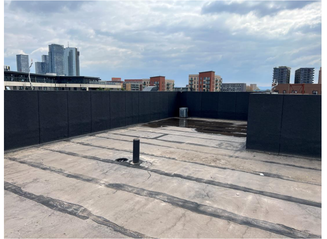
Block B main roof covering preparation
