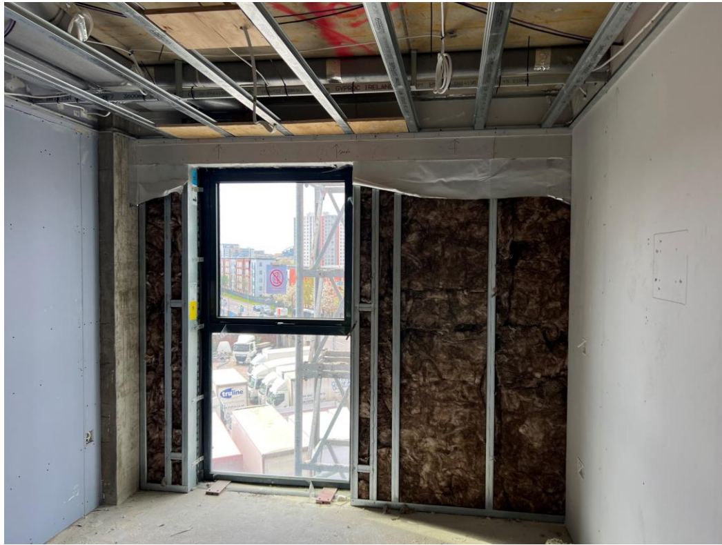
Level 4 – walls insulated ready for boarding
