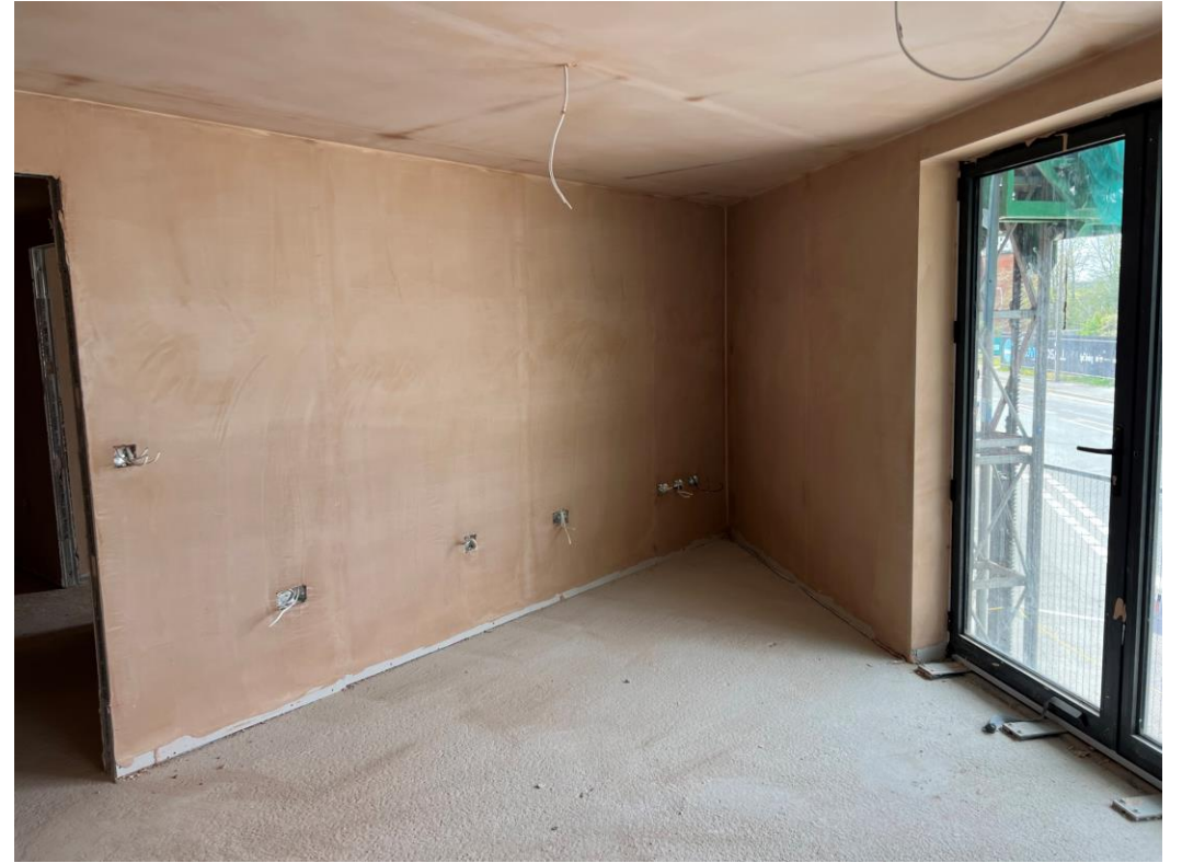
Level 1 – walls and ceilings plastered
