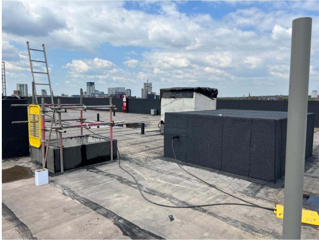
Block B main roof covering preparation
