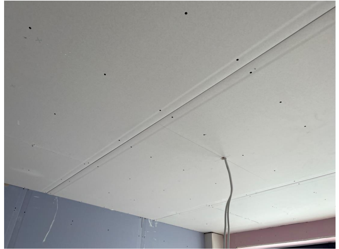
Level 2 – ceilings boarded
