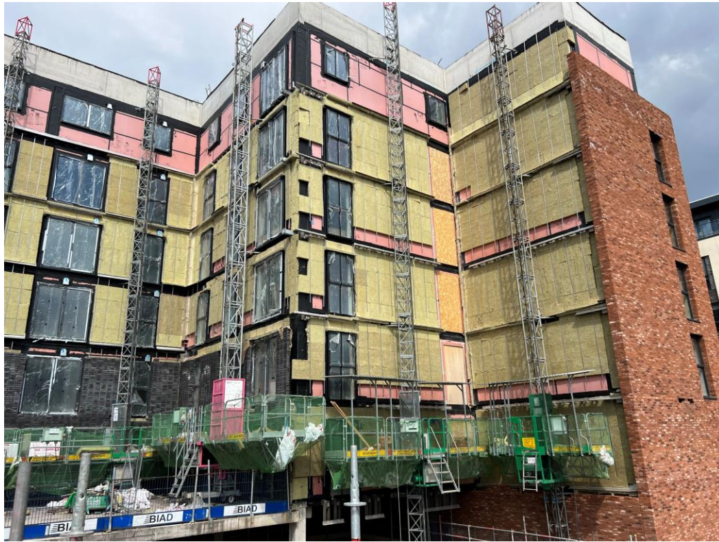
Block B wall insulation & brickwork
