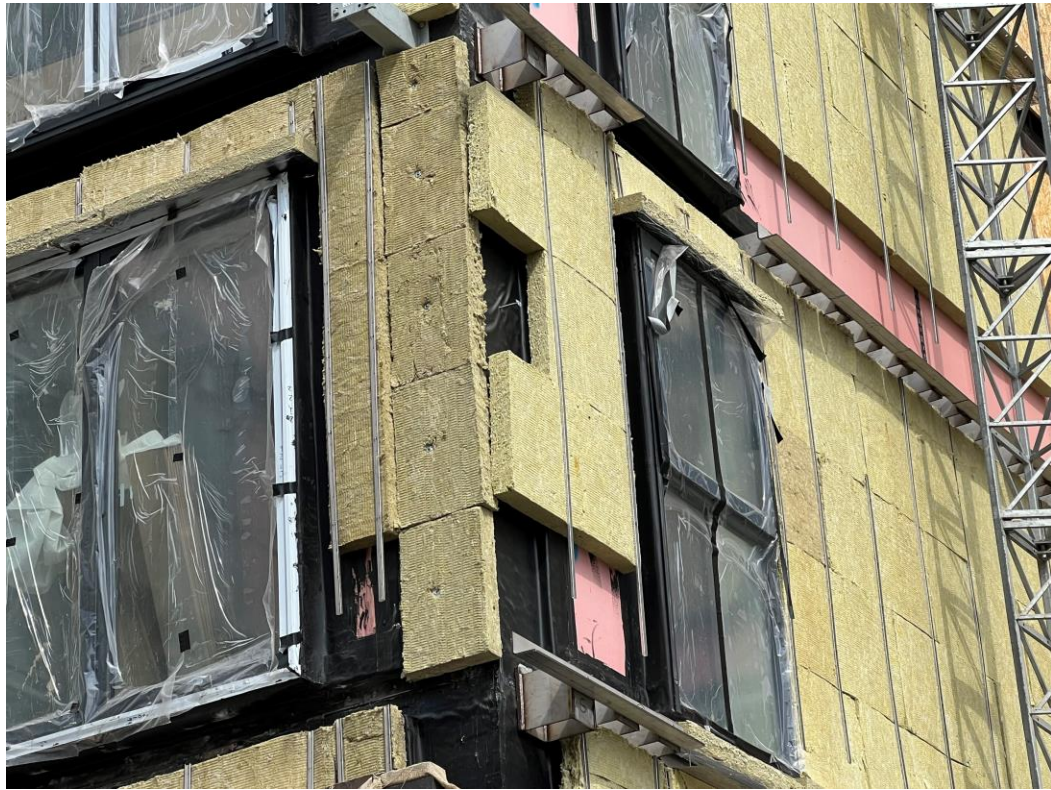
Block B masonry support
