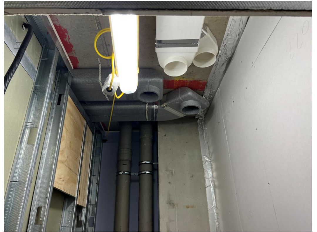
Ground floor Apartments 1 st fix mechanical
