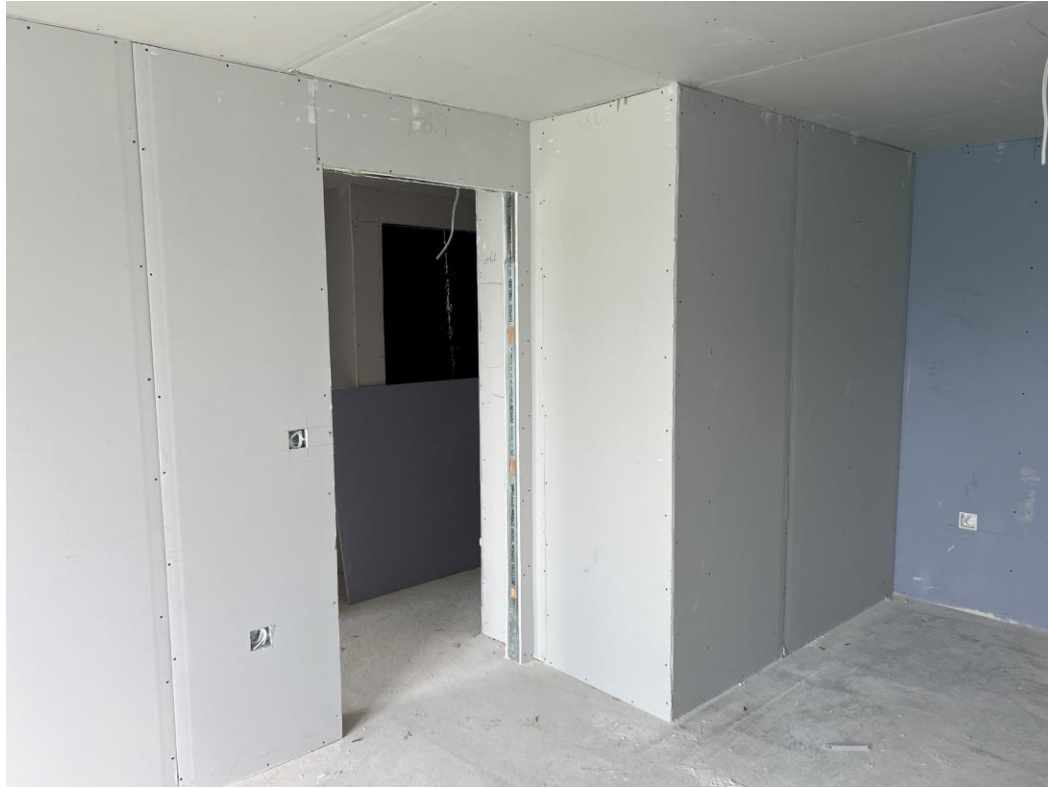
Level 2 – ceilings boarded
