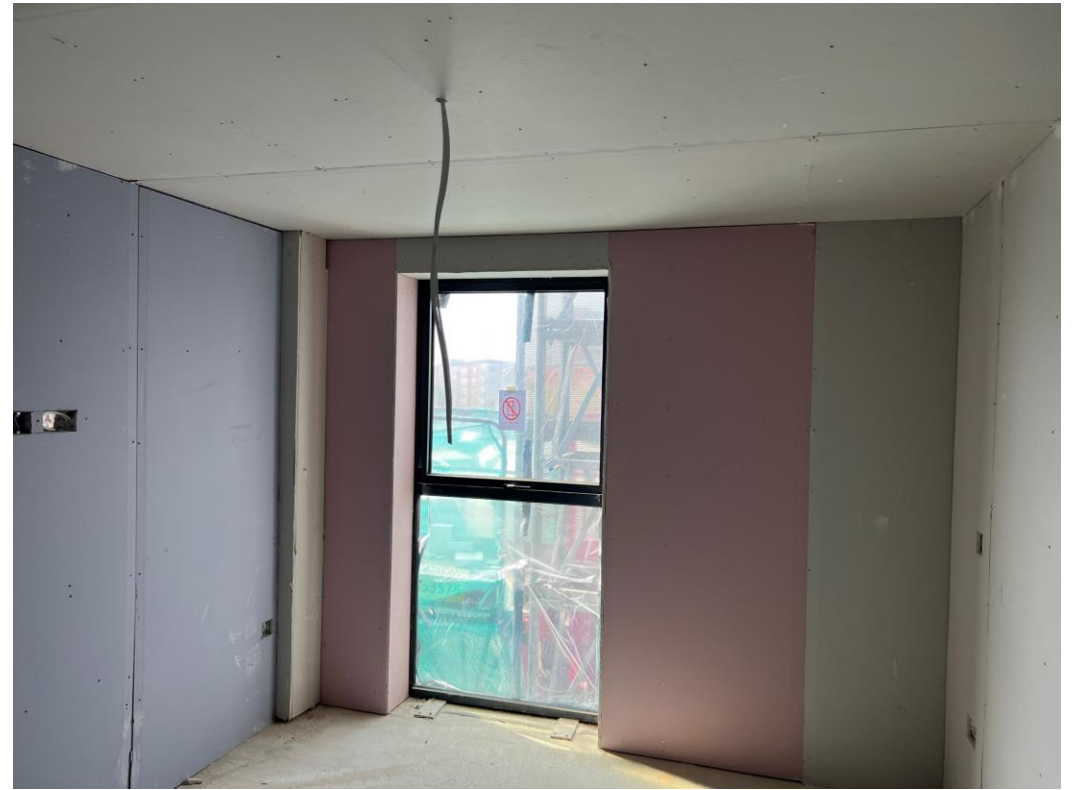
Level 2 – ceilings boarded
