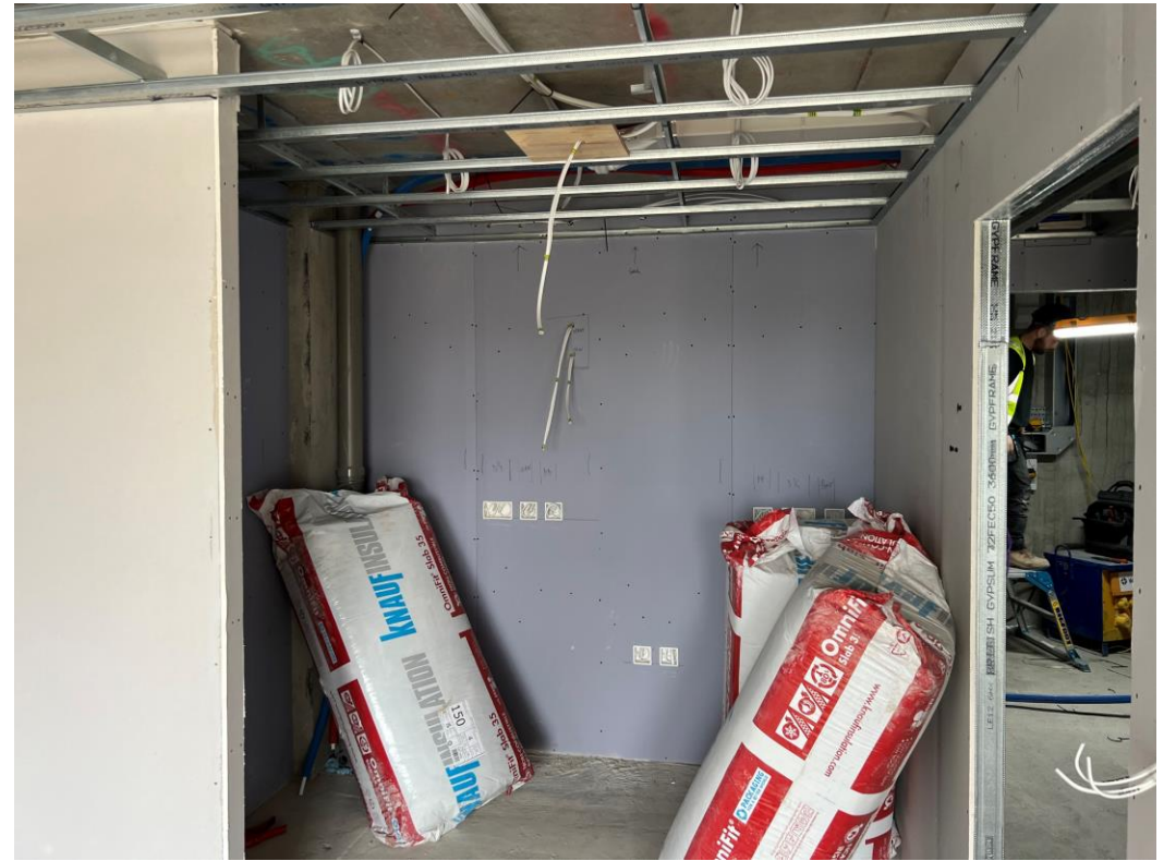
Level 5 – ceiling installation
