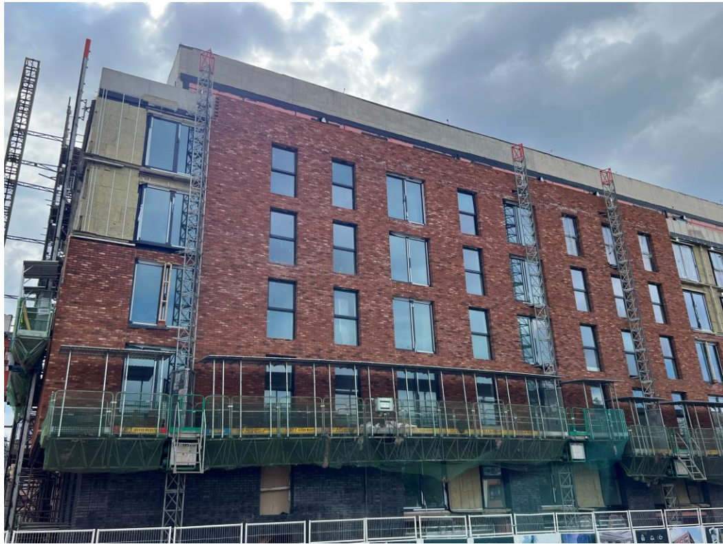
Ordsall Lane site view
