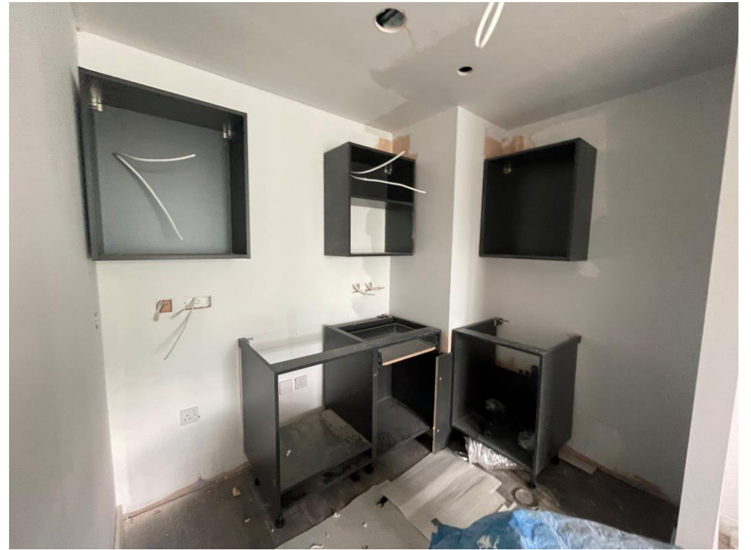
Kitchen units commenced
