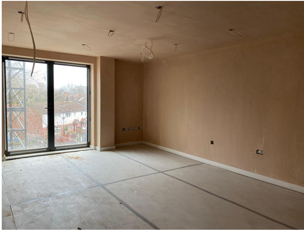
Doorframes, skirting and architrave
