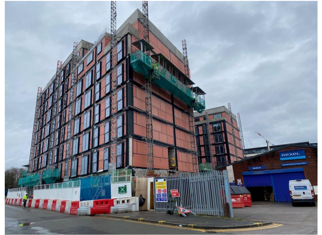
Worrall Street site view
