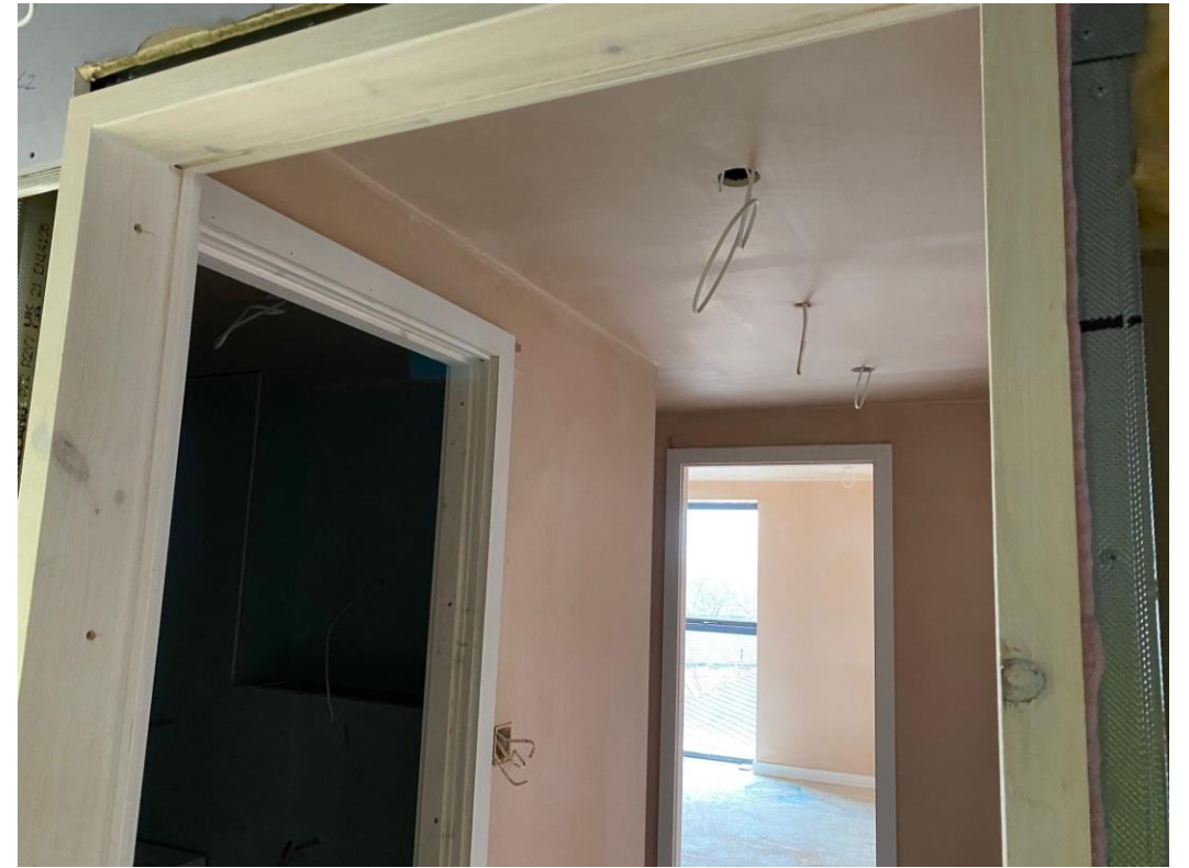
Doorframes, skirting and architrave
