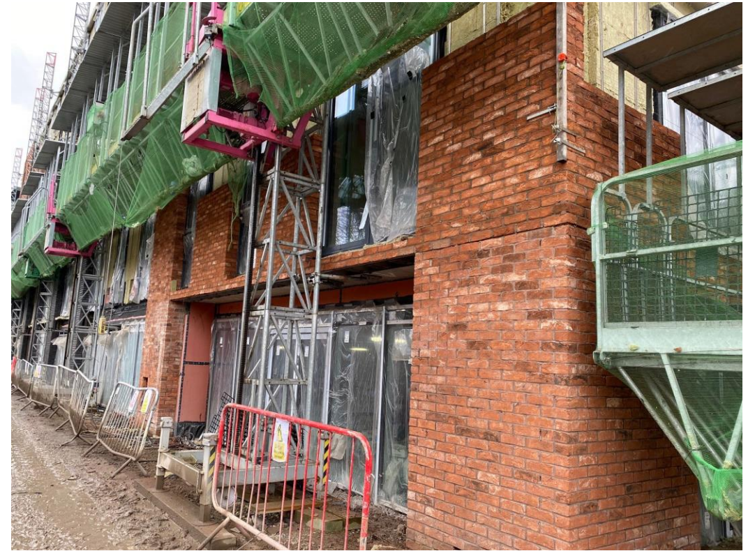
Block B wall insulation & brickwork
