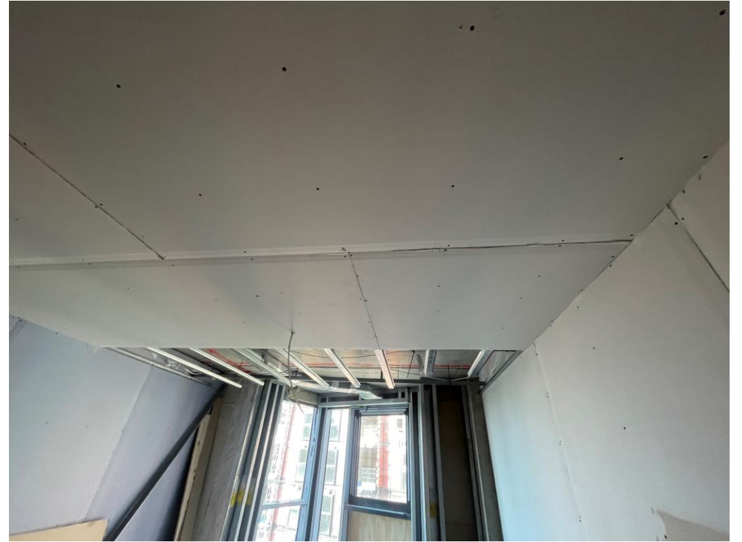
Partition walls and ceiling
