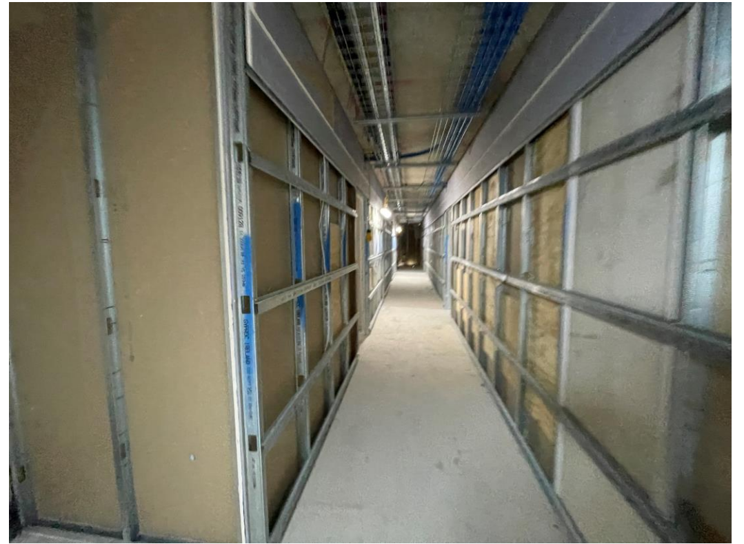
Partition walls forming apartments
