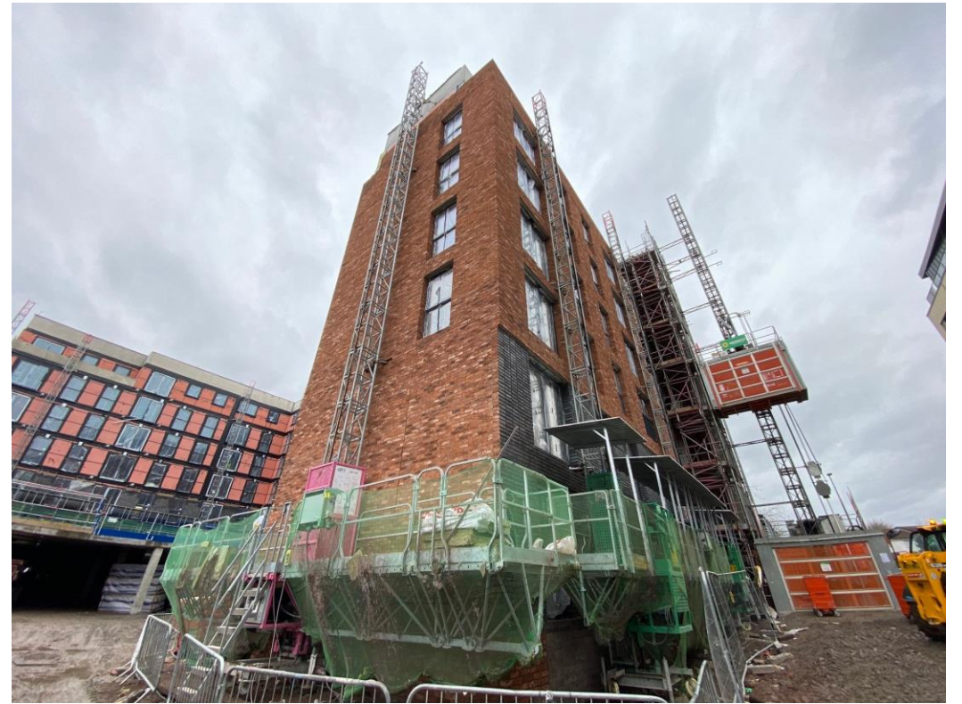
Block B facing brickwork
