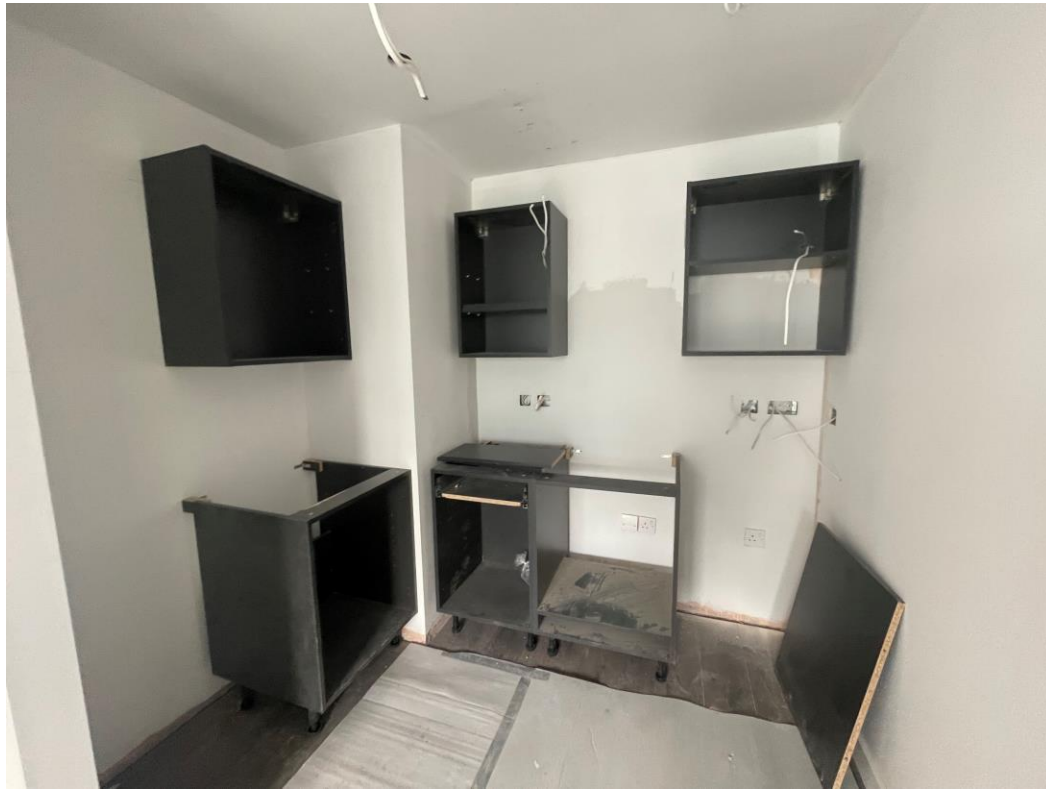
Kitchen units commenced
