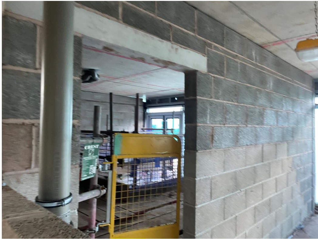
Ground level walls formed
