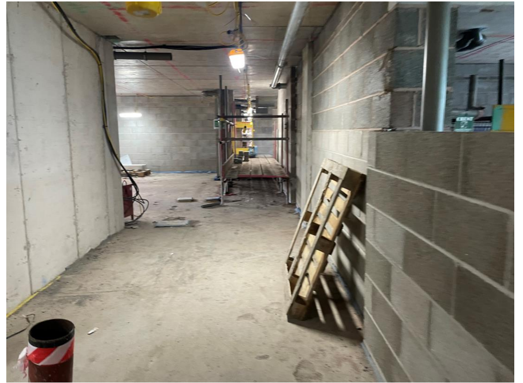
Ground level walls formed
