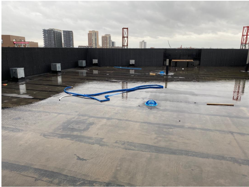
Block B terrace roof covering preparation
