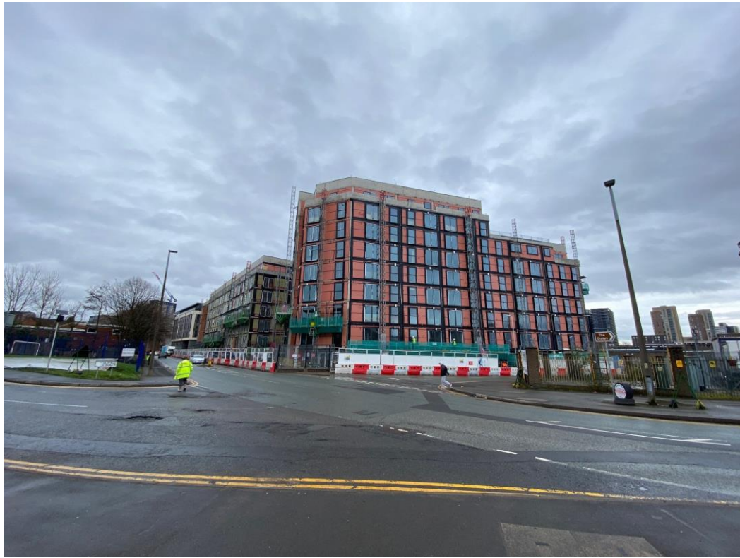
Ordsall Lane site view
