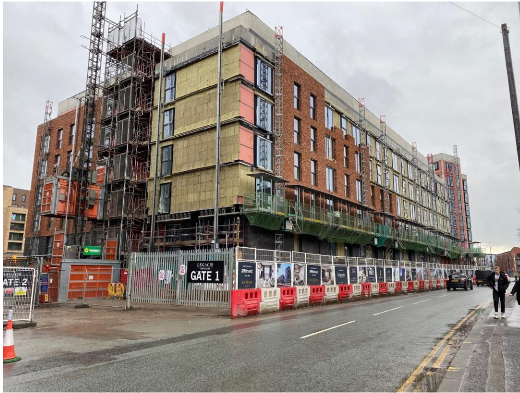
Ordsall Lane site view
