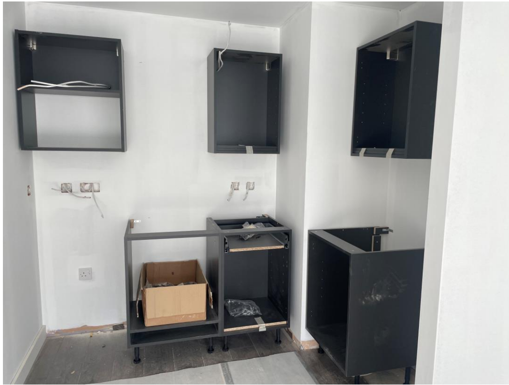
Kitchen units commenced
