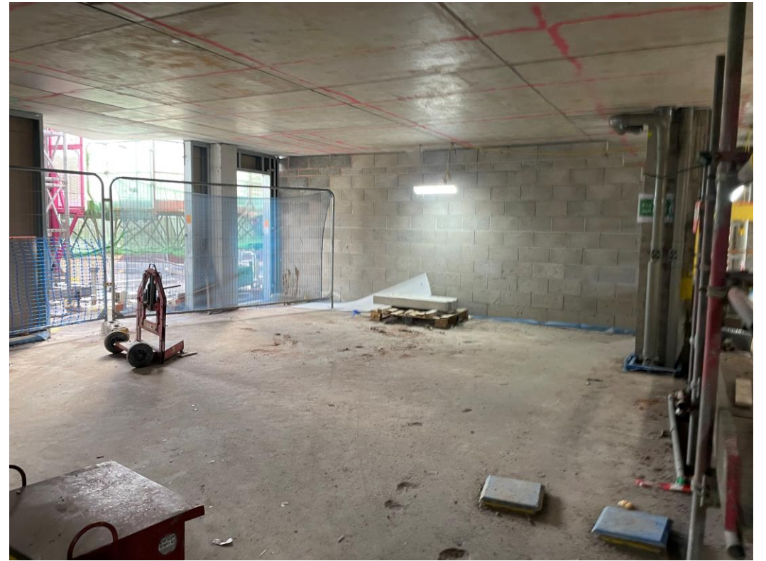
Ground level walls formed
