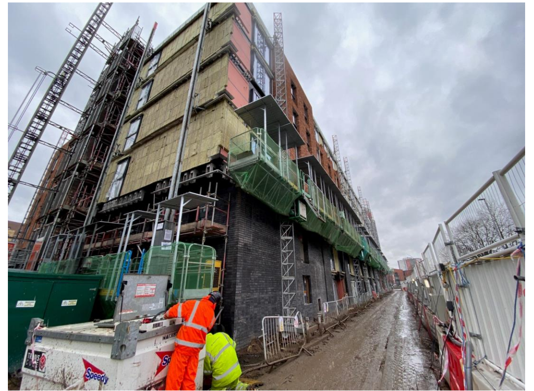
Block B wall insulation & brickwork
