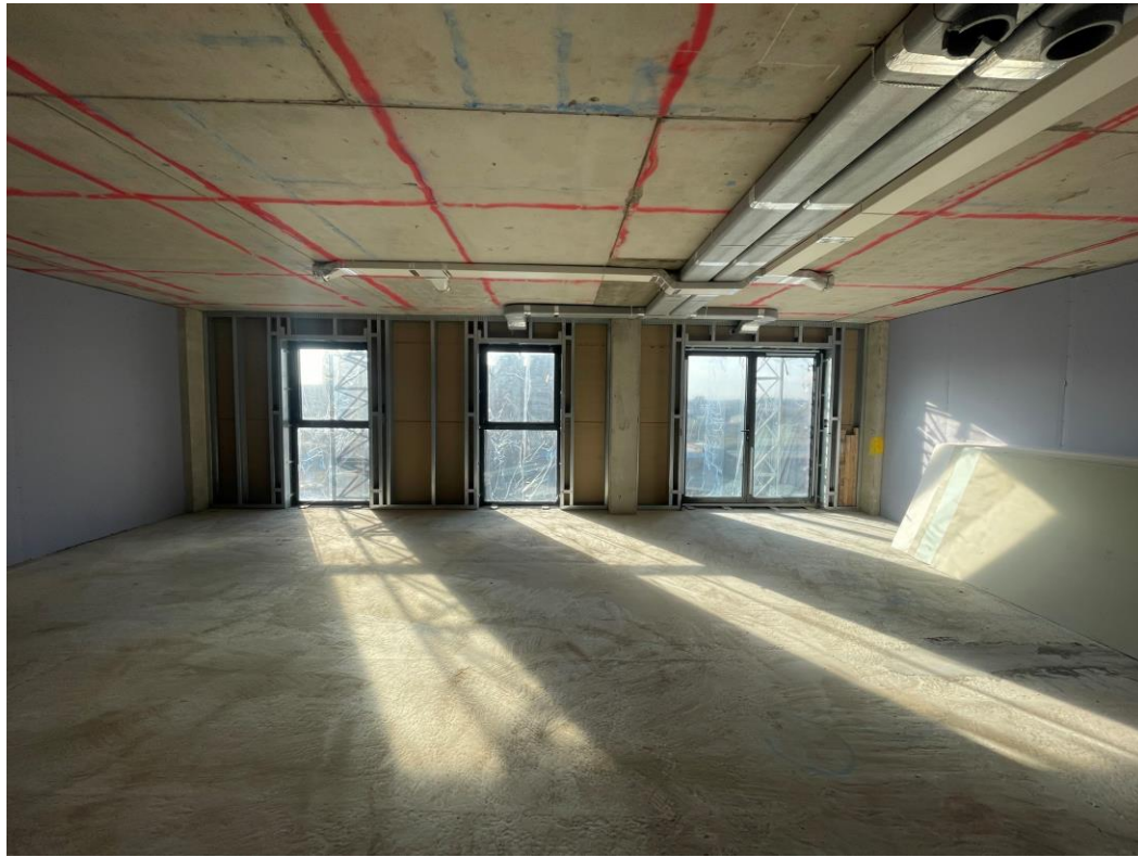
Upper floor mechanical services ongoing
