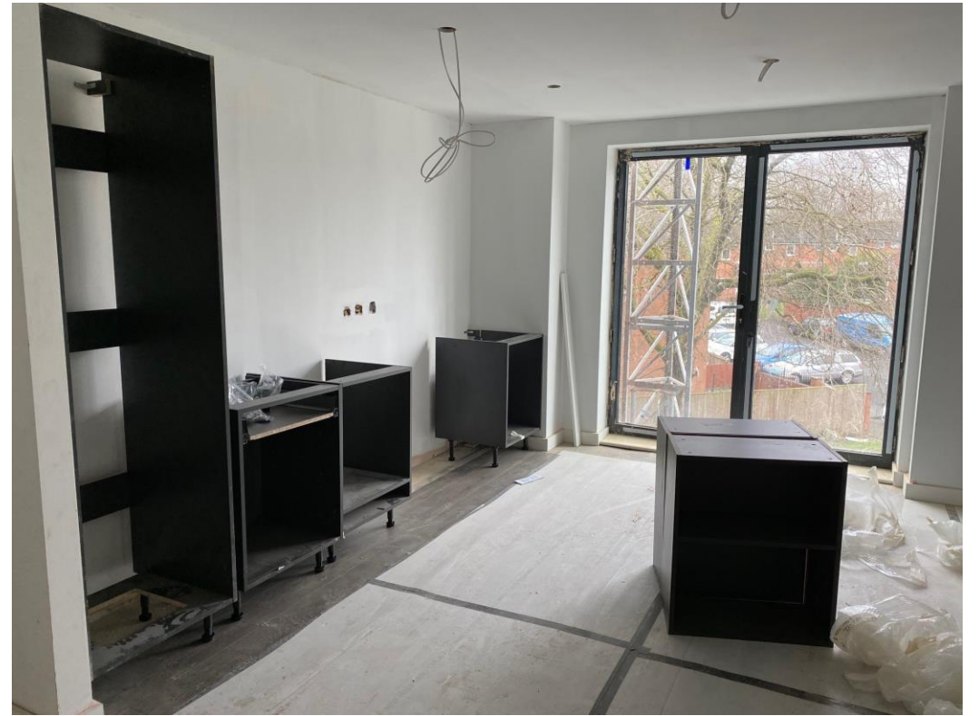
Kitchen units commenced
