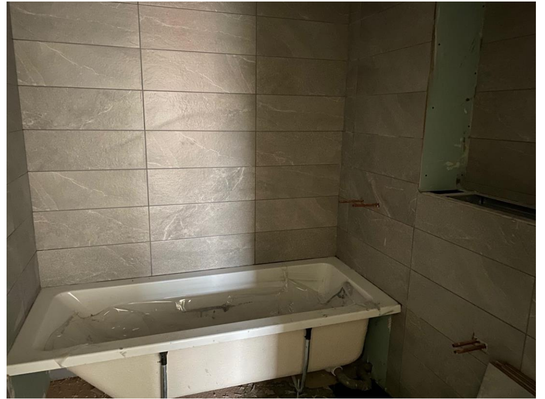
Wall and floor tiling ongoing
