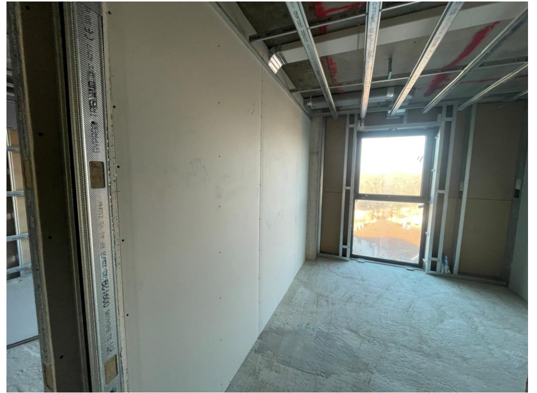
Partition walls and ceiling
