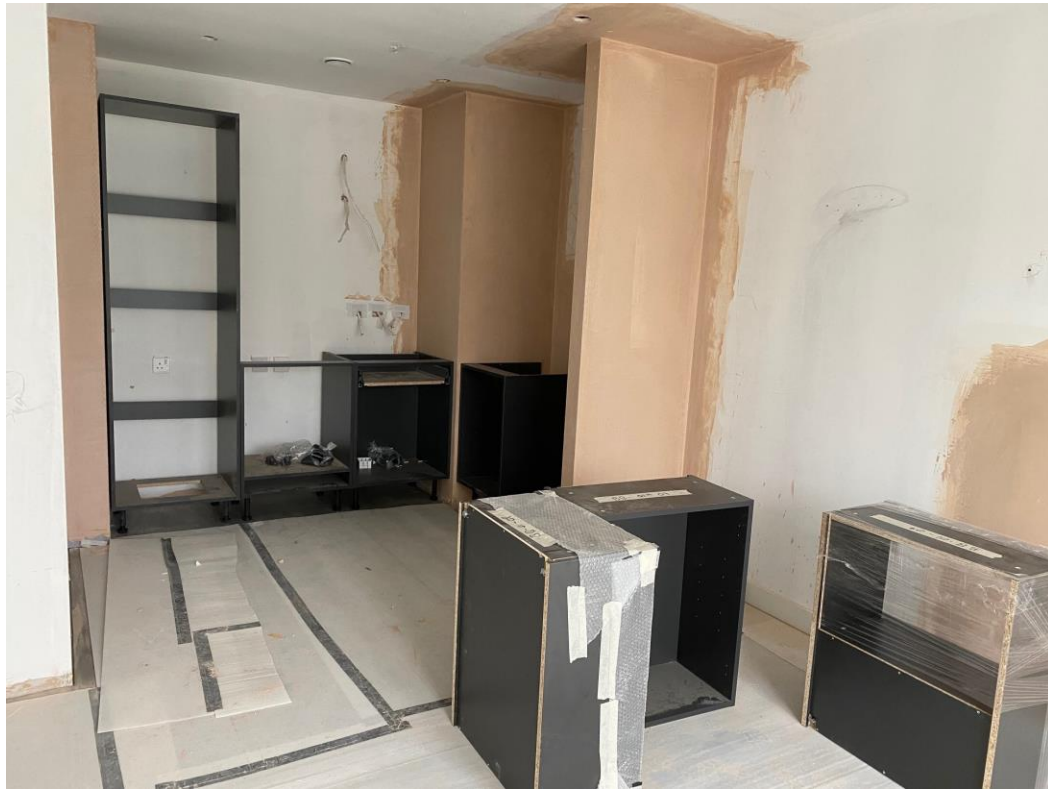
Kitchen units commenced
