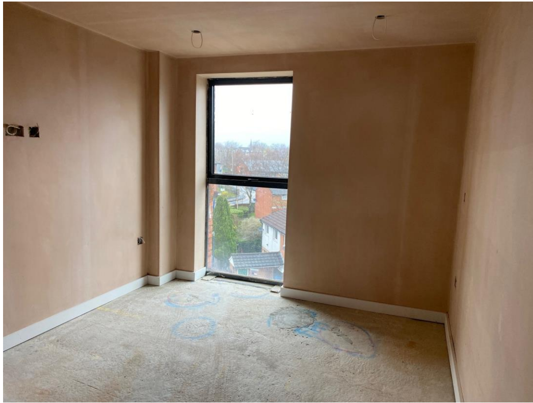
Doorframes, skirting and architrave
