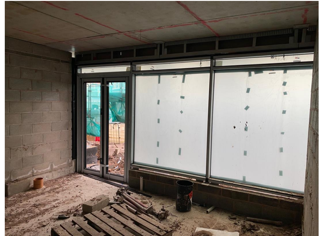
Ground floor curtain wall frame & glazing installed
