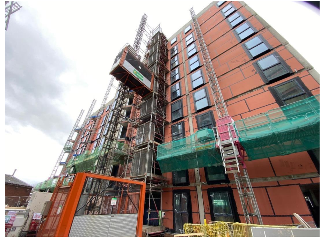
Block A weatherboarding & windows installed
