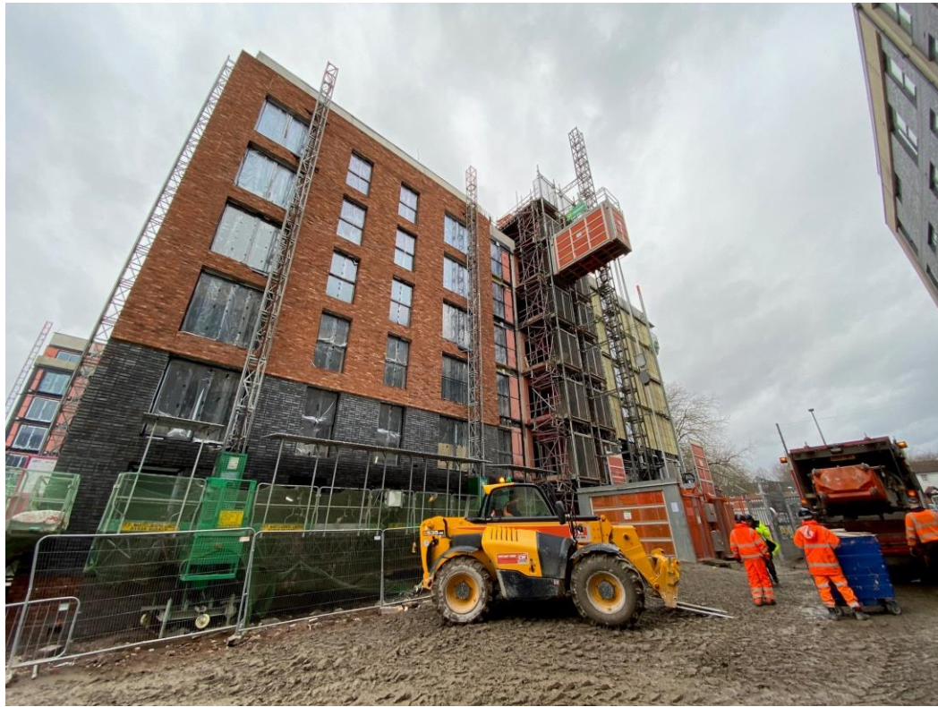
Block B wall insulation & brickwork
