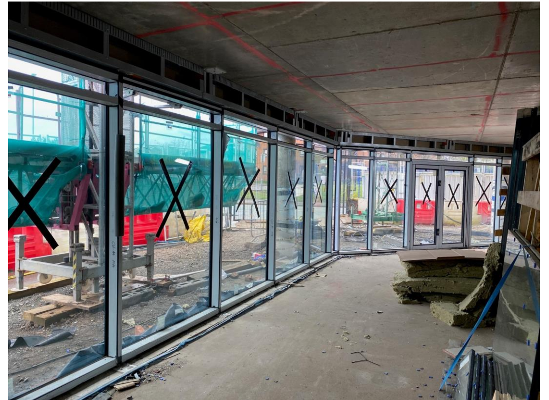
Ground floor curtain wall frame & glazing installed
