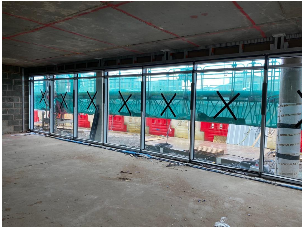
Ground floor curtain wall frame & glazing installed
