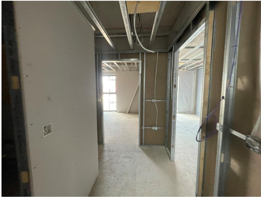
Partition walls and ceiling
