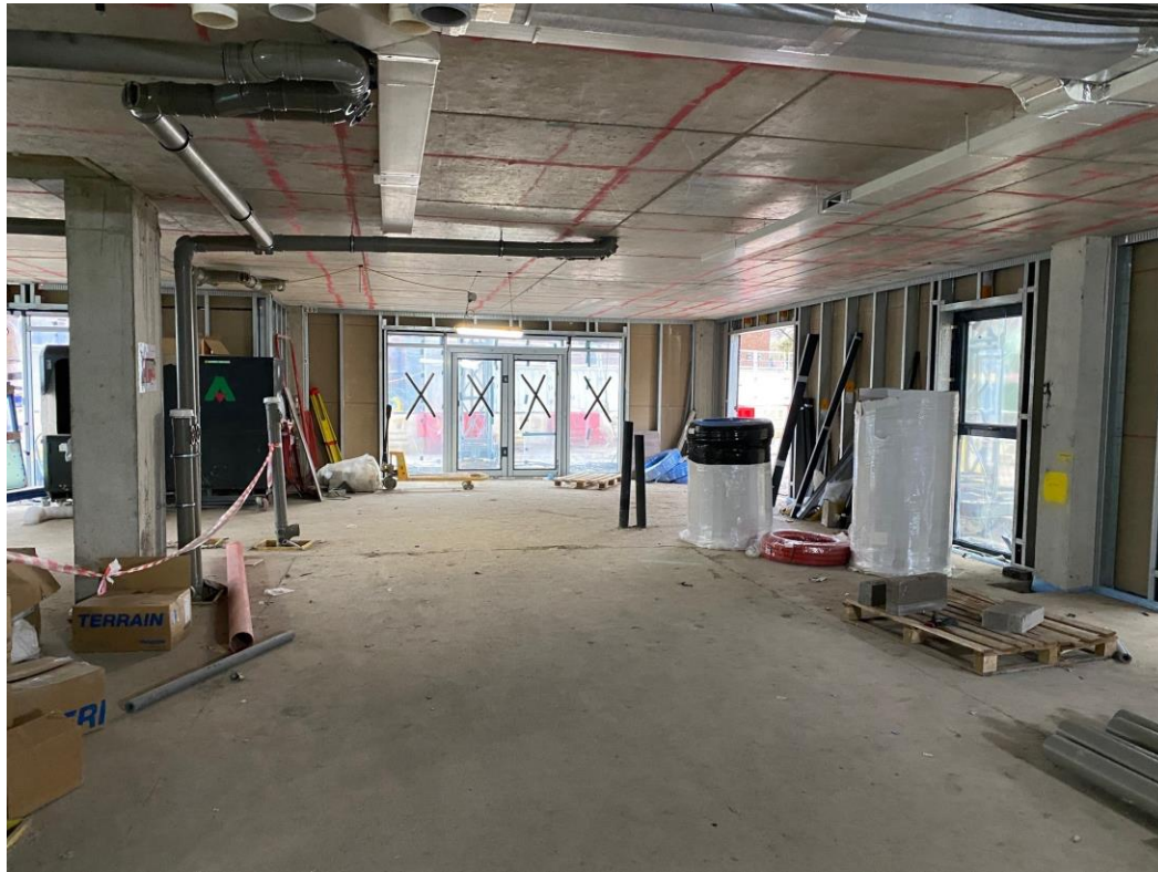
Ground floor curtain wall frame & glazing installed
