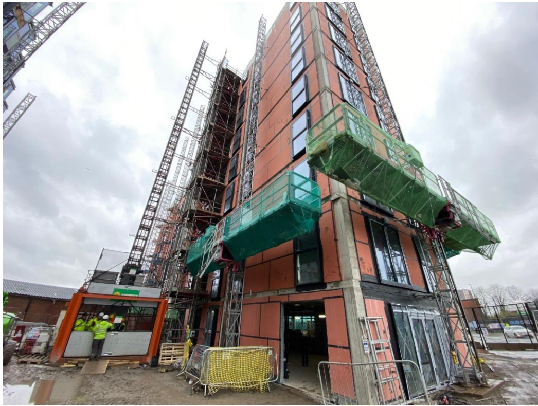
Block A weatherboarding & windows installed
