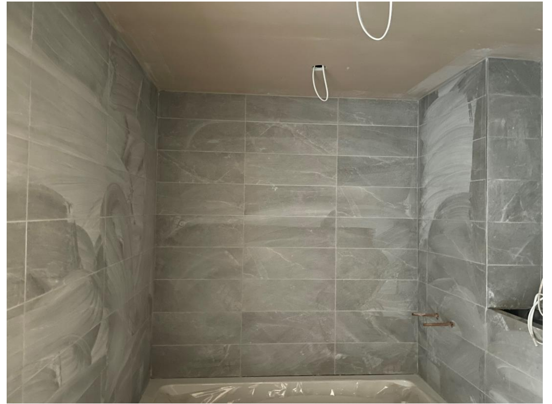
Wall and floor tiling ongoing
