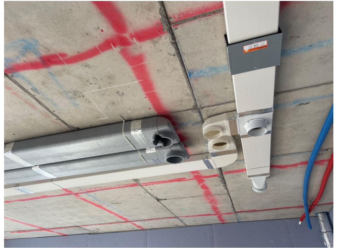
Upper floor mechanical services ongoing
