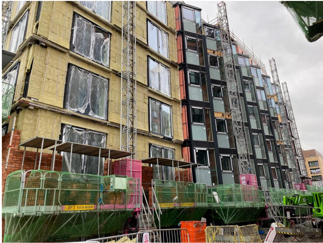
Block B wall insulation & brickwork
