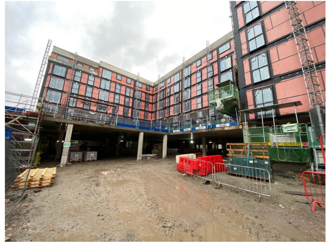
Block B wall preparation for insulation & brickwork
