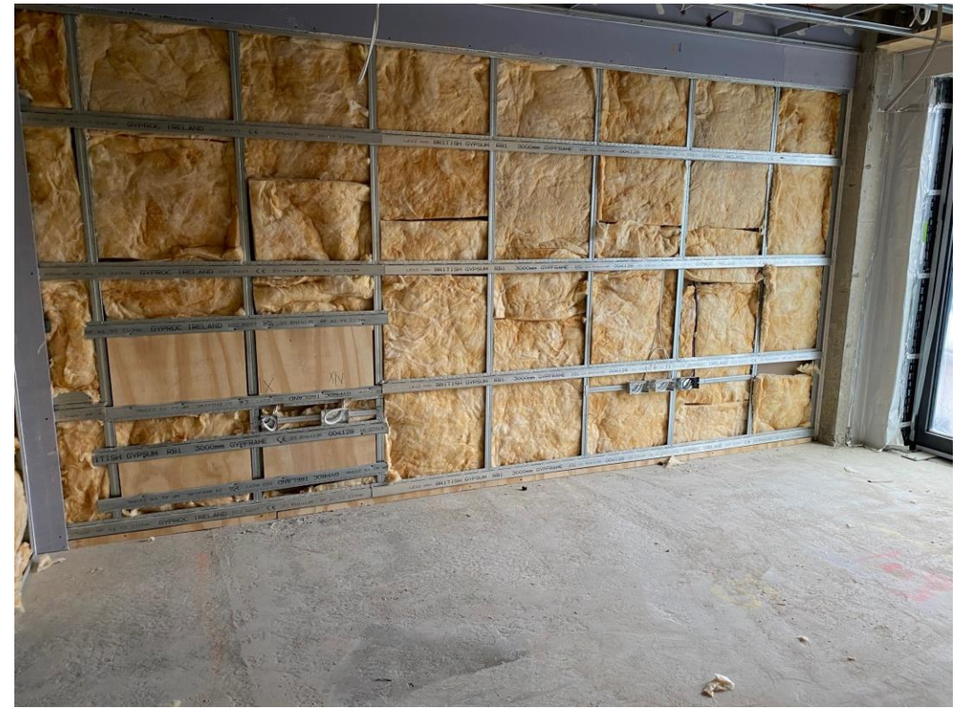
Partition walls forming apartments
