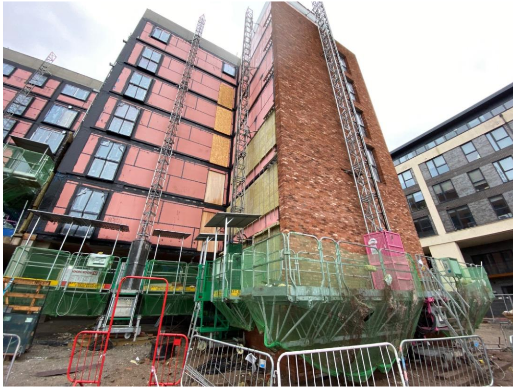
Block B wall insulation & brickwork
