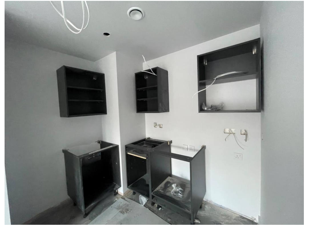
Kitchen units commenced
