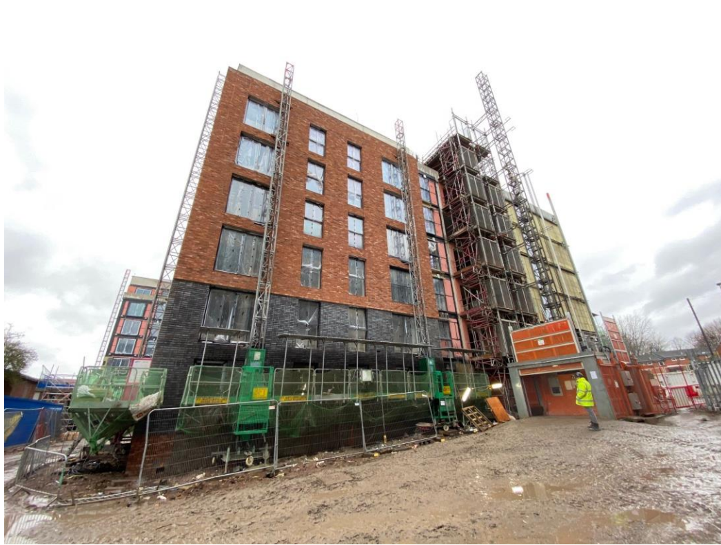
Block B wall insulation & brickwork
