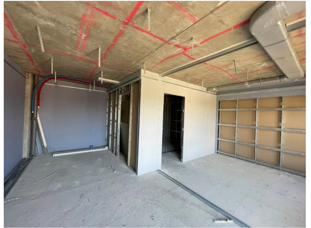
Partition wall setting out
