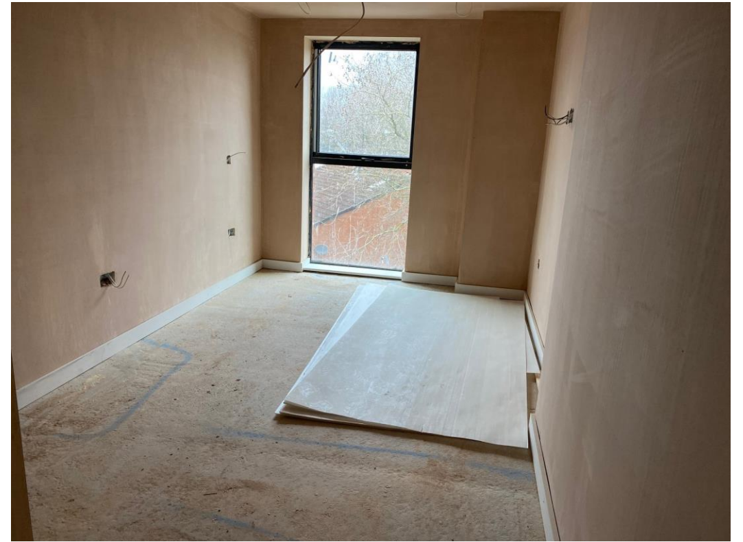
Doorframes, skirting and architrave
