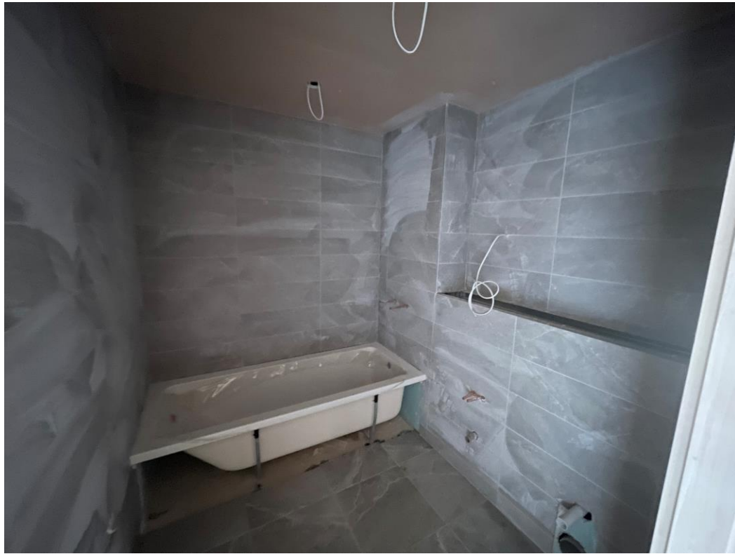
Wall and floor tiling ongoing
