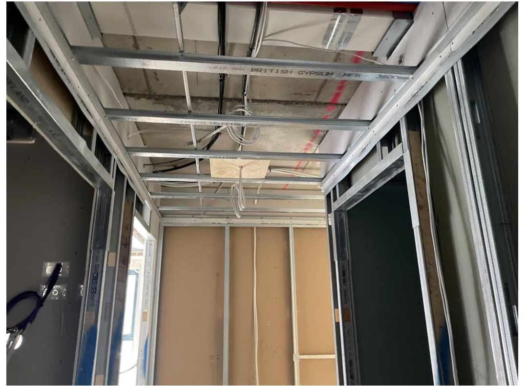
Partition walls and ceiling
