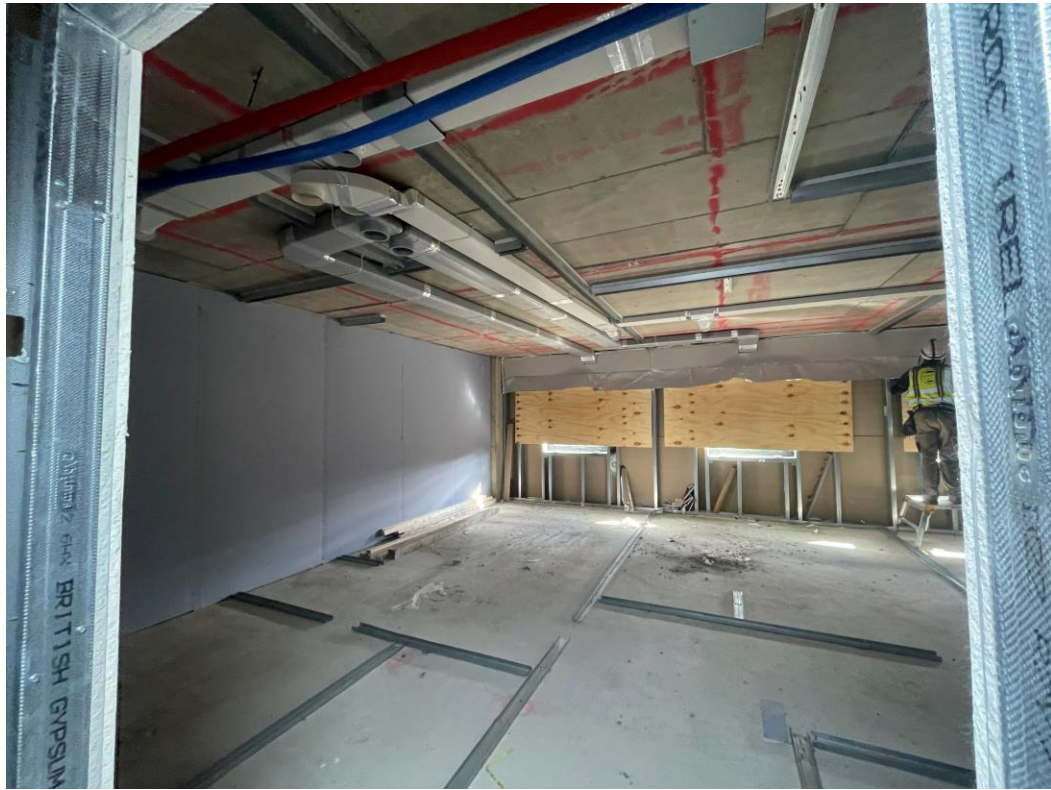
Partition wall setting out
