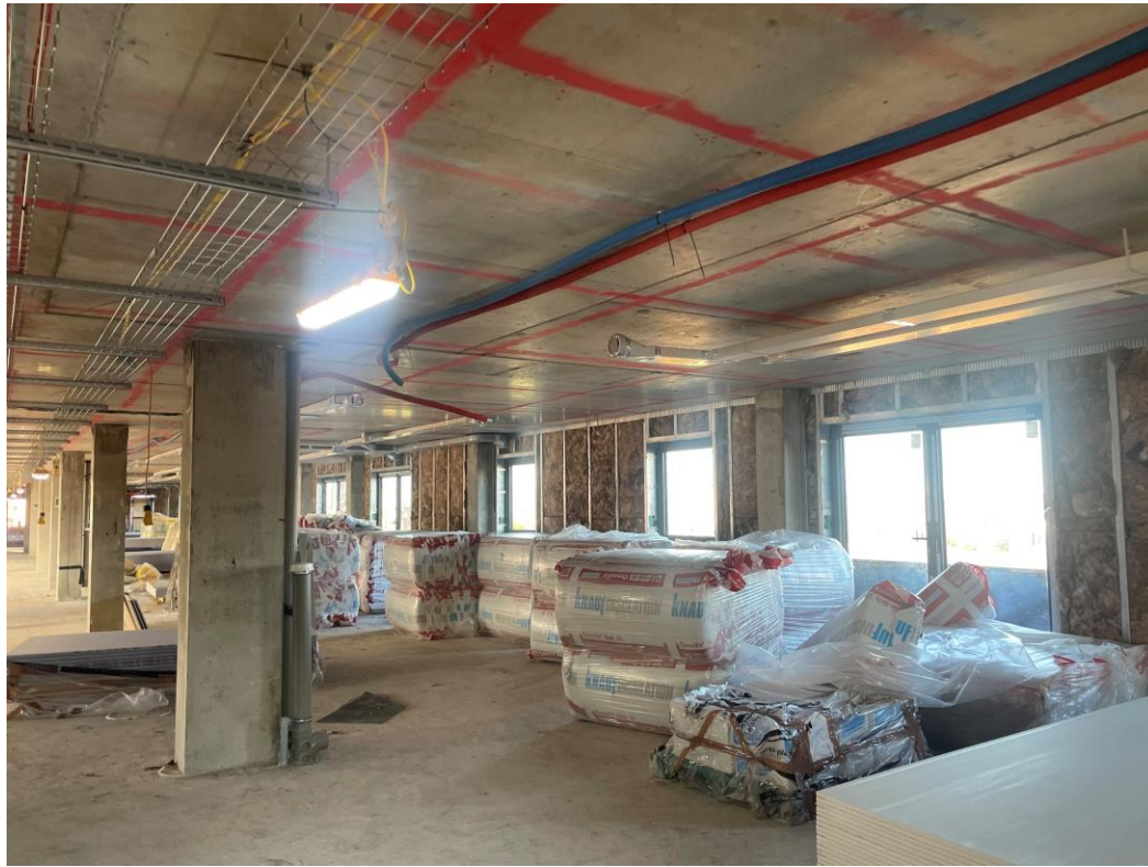
External walls upper floor levels to receive insulation & boarding
