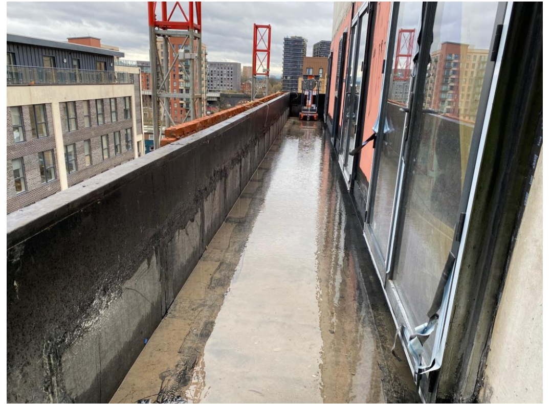
Block B balcony roof covering preparation
