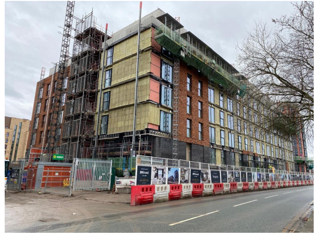
Ordsall Lane site view
