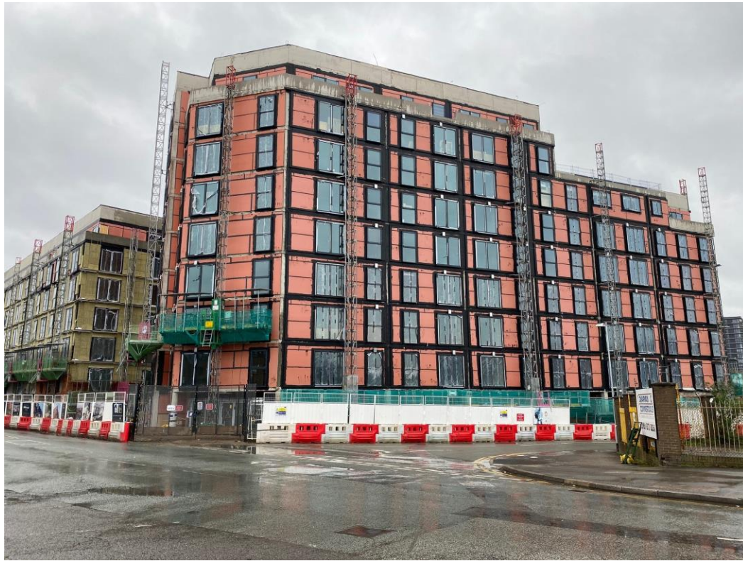
Ordsall Lane site view
