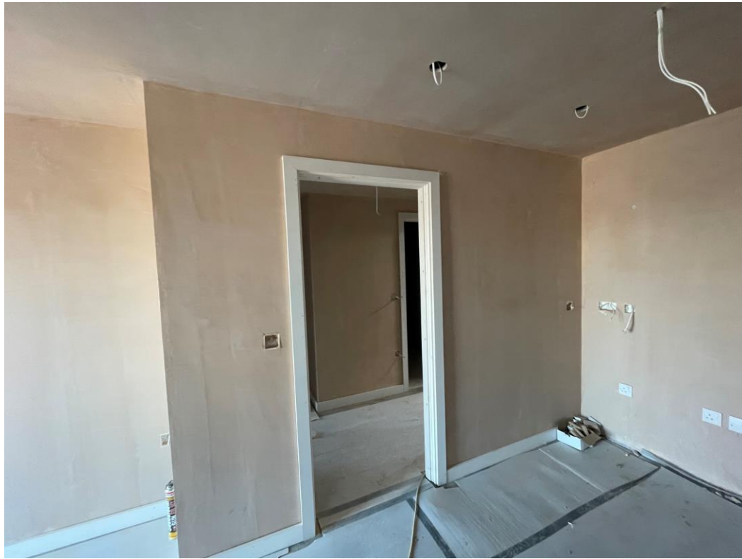
Doorframes, skirting and architrave
