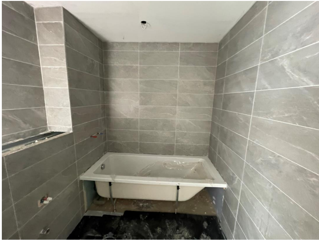
Wall and floor tiling ongoing
