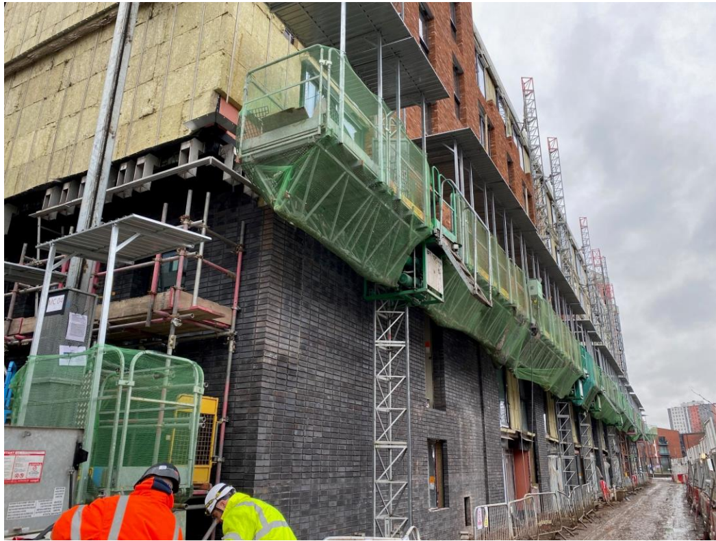
Block B wall insulation & brickwork
