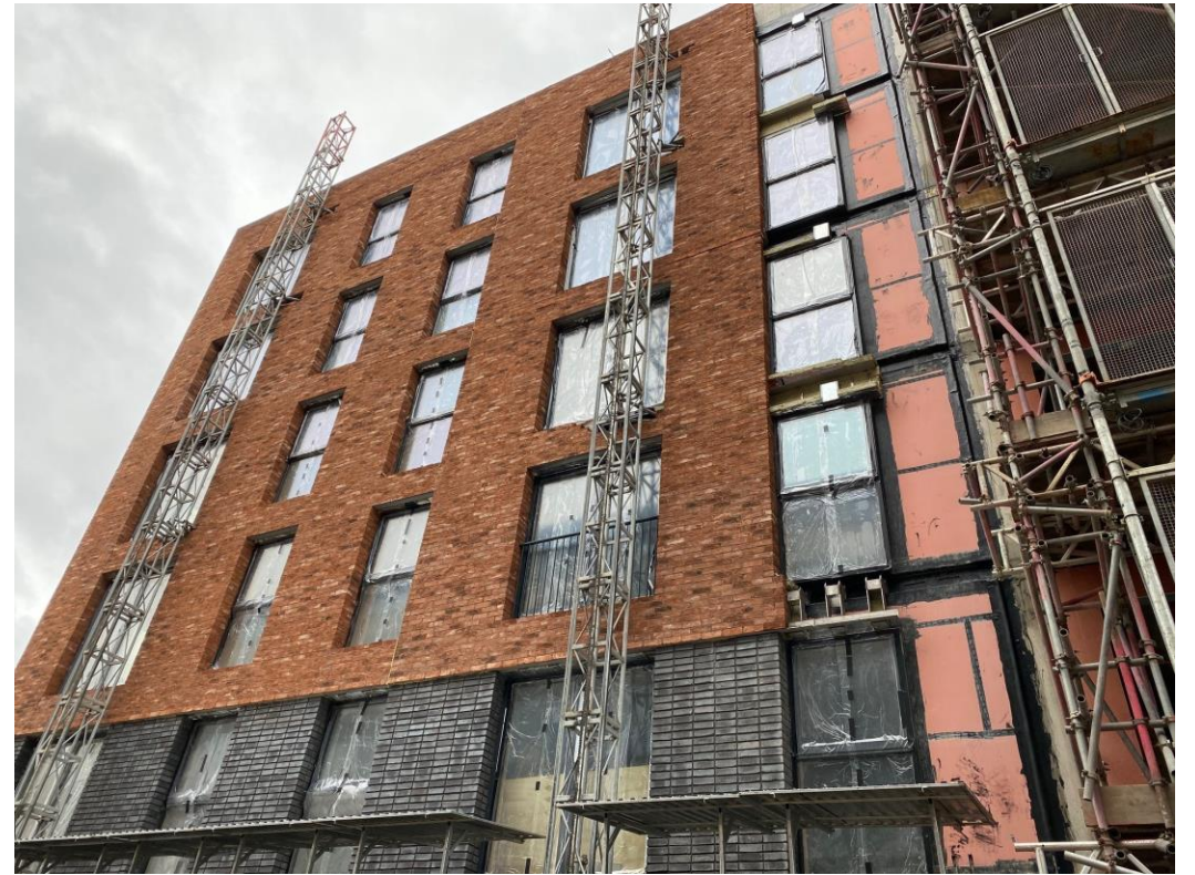
Block B facing brickwork
