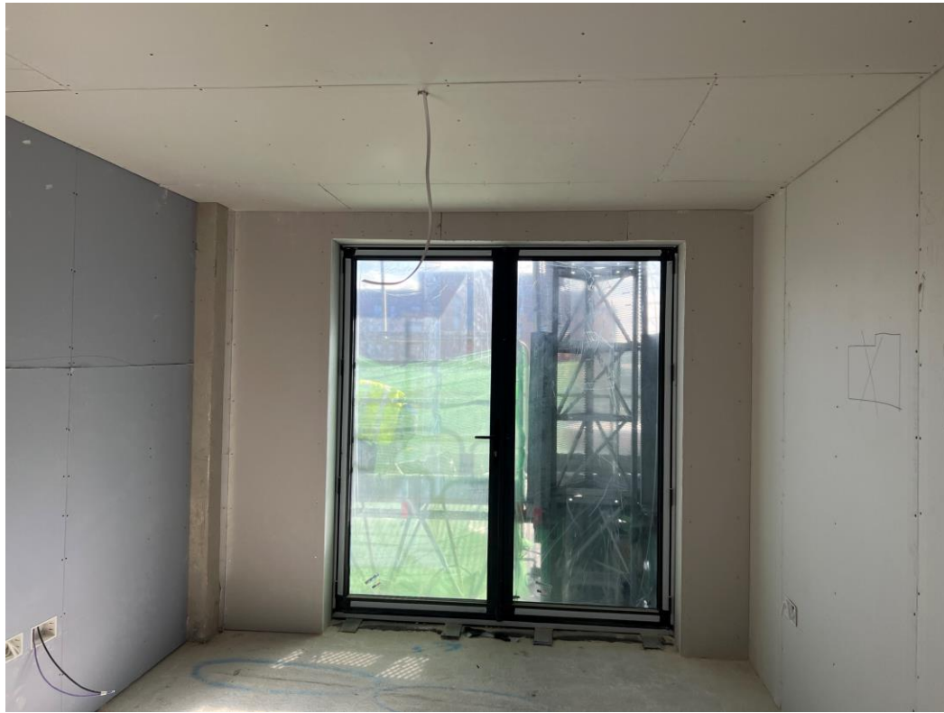
Apartment ready for plaster skim
