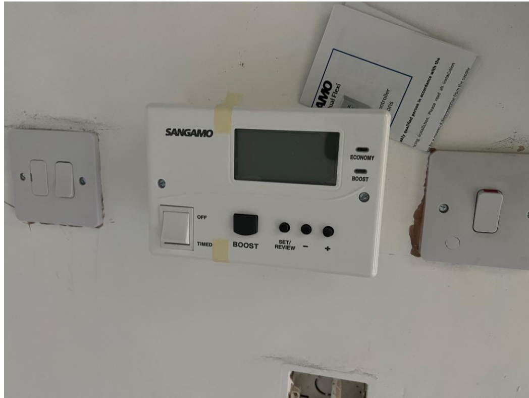
2 nd fix electrical
