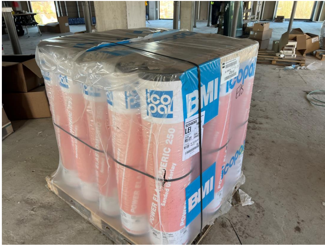
Block A roof materials
