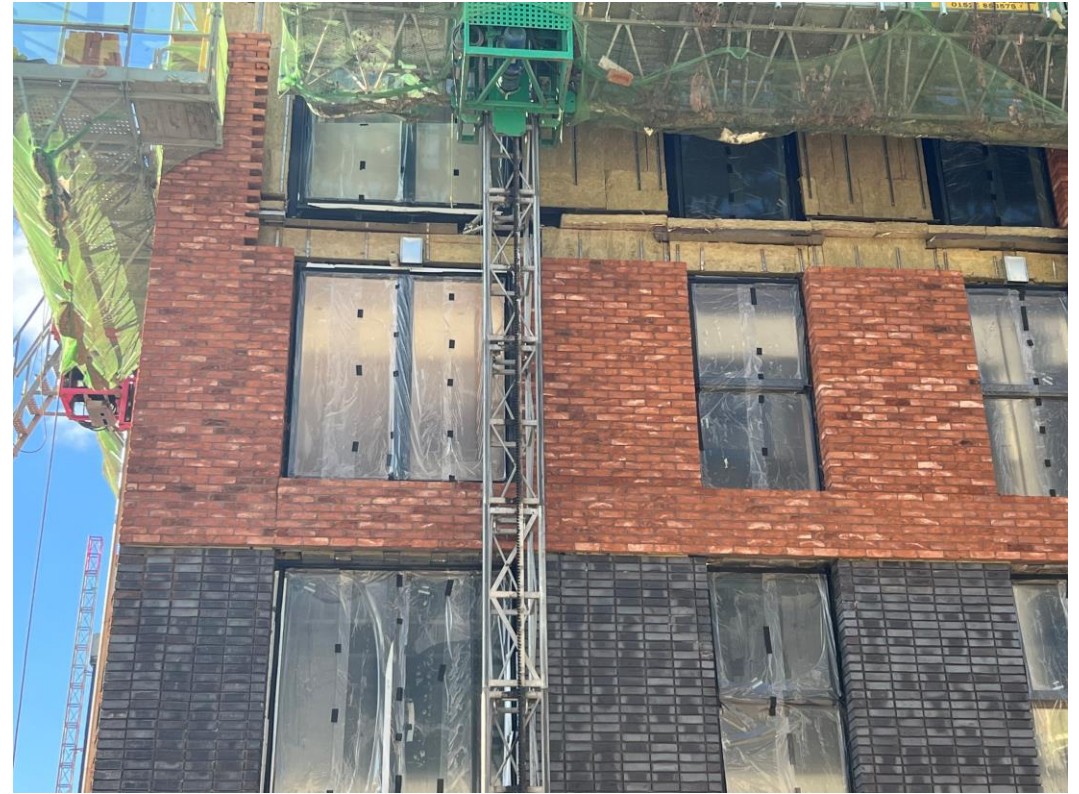
Block B facing brickwork
