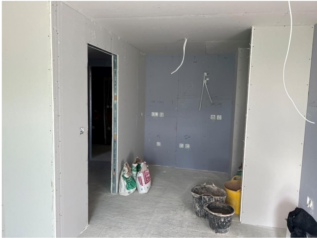
Apartment 1 st fix electrical
