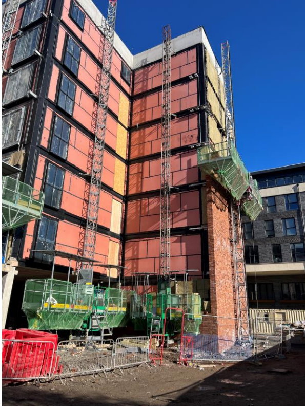
Block B facing brickwork
