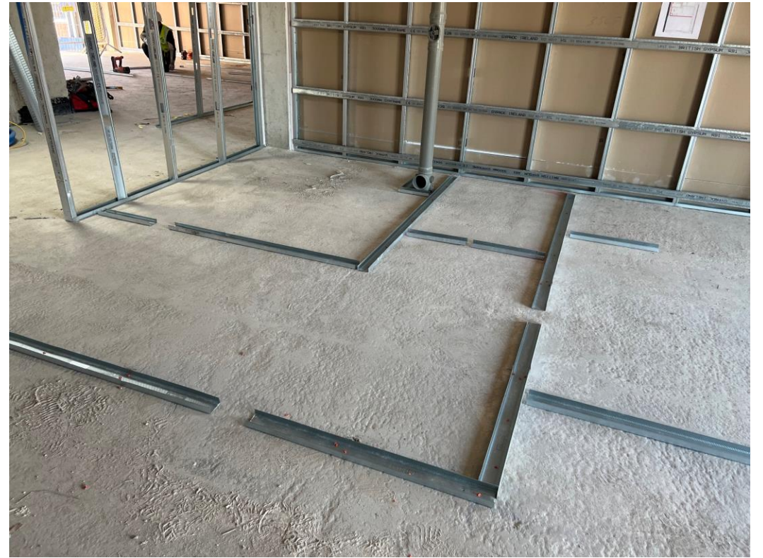
3 rd Floor partition walls
