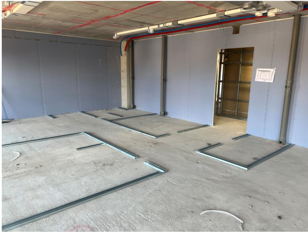
3 rd Floor partition walls
