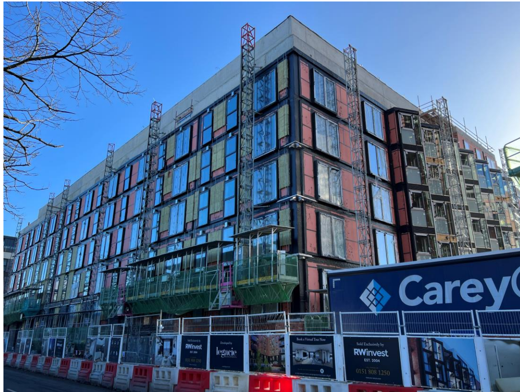
Ordsall Lane site view
