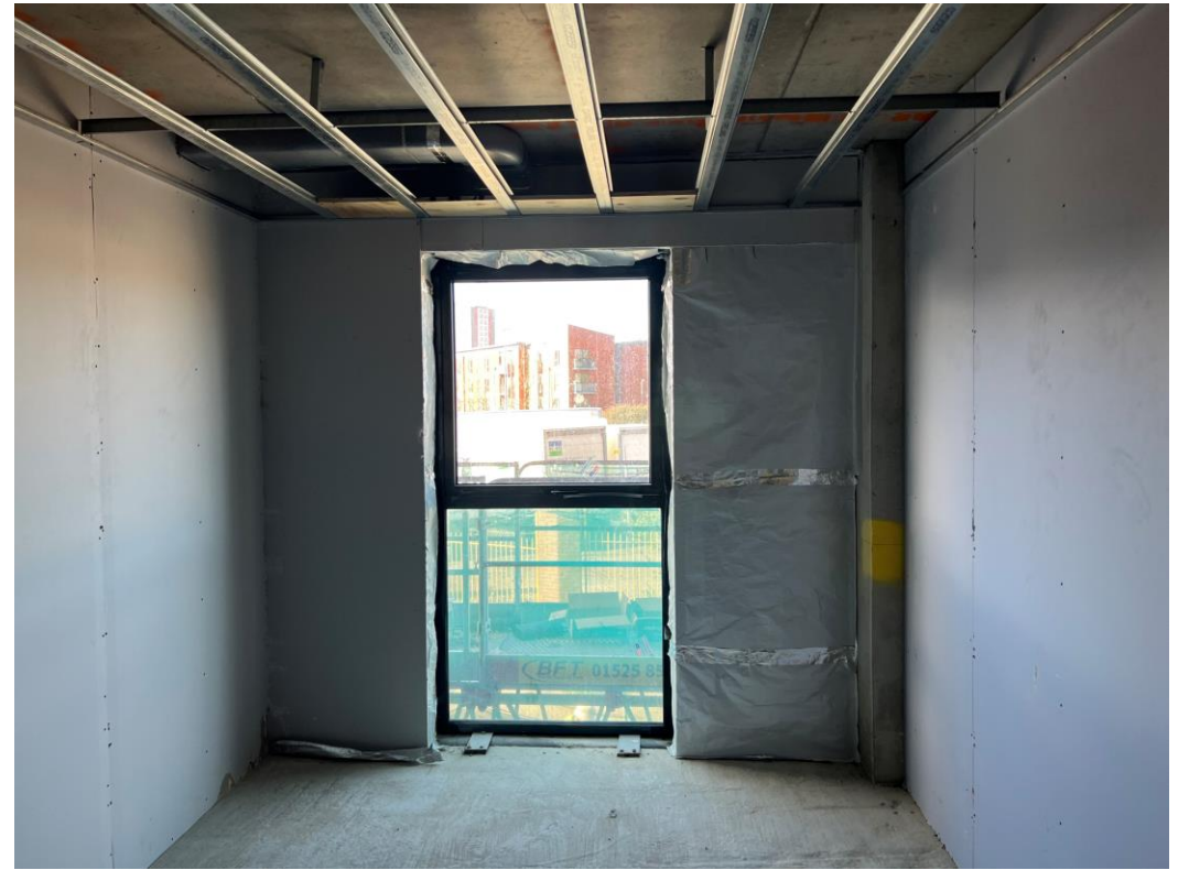
1 st Floor partition walls and ceiling
