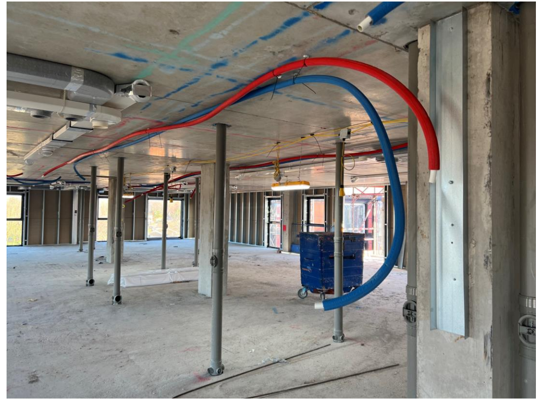
Upper level 1 st fix mechanical ducting & water
