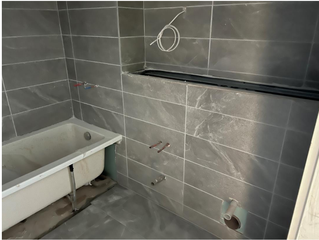
Wall and floor tiling commenced
