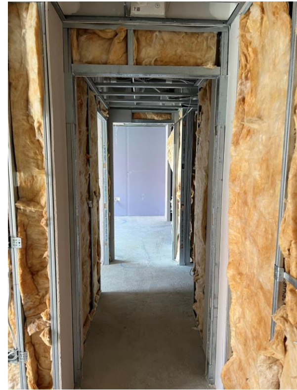
Upper floor Apartment partitions ongoing
