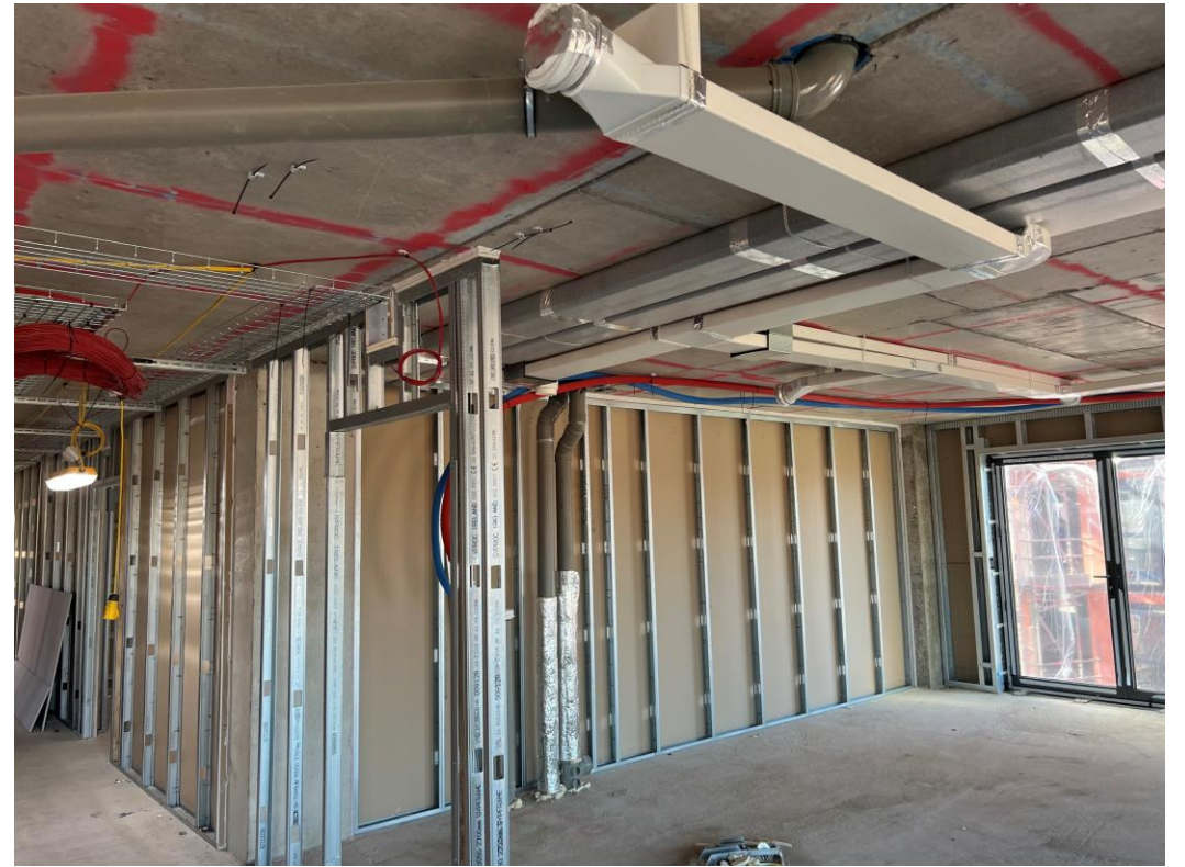
Upper floor Apartment partitions ongoing
