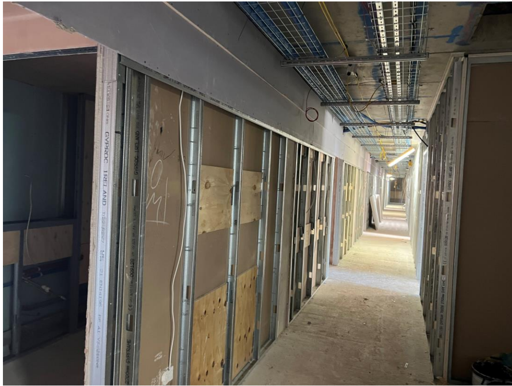
Upper floor Apartment partitions ongoing
