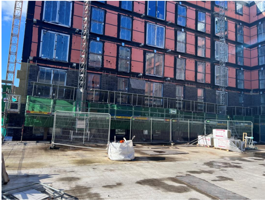
Block B Podium facing brickwork
