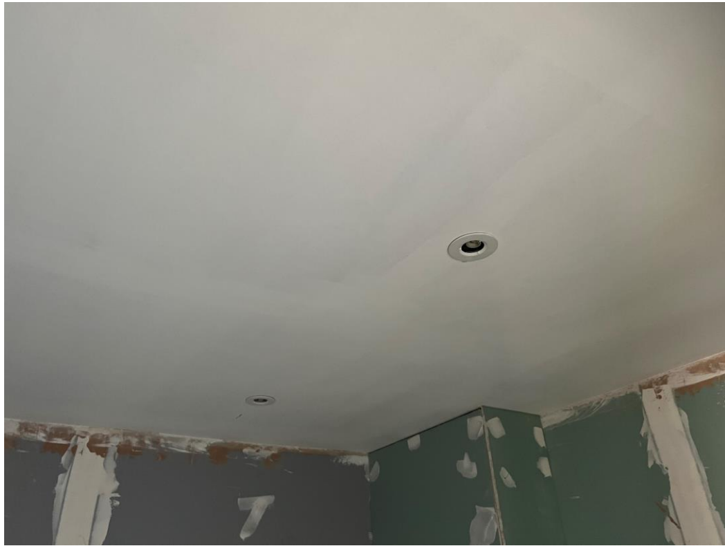
2 nd fix electrical
