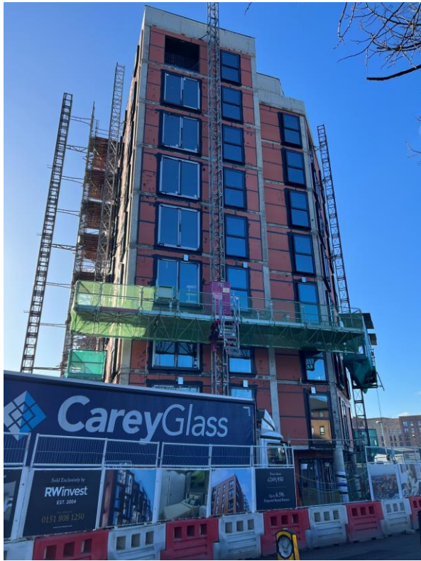
Ordsall Lane site view
