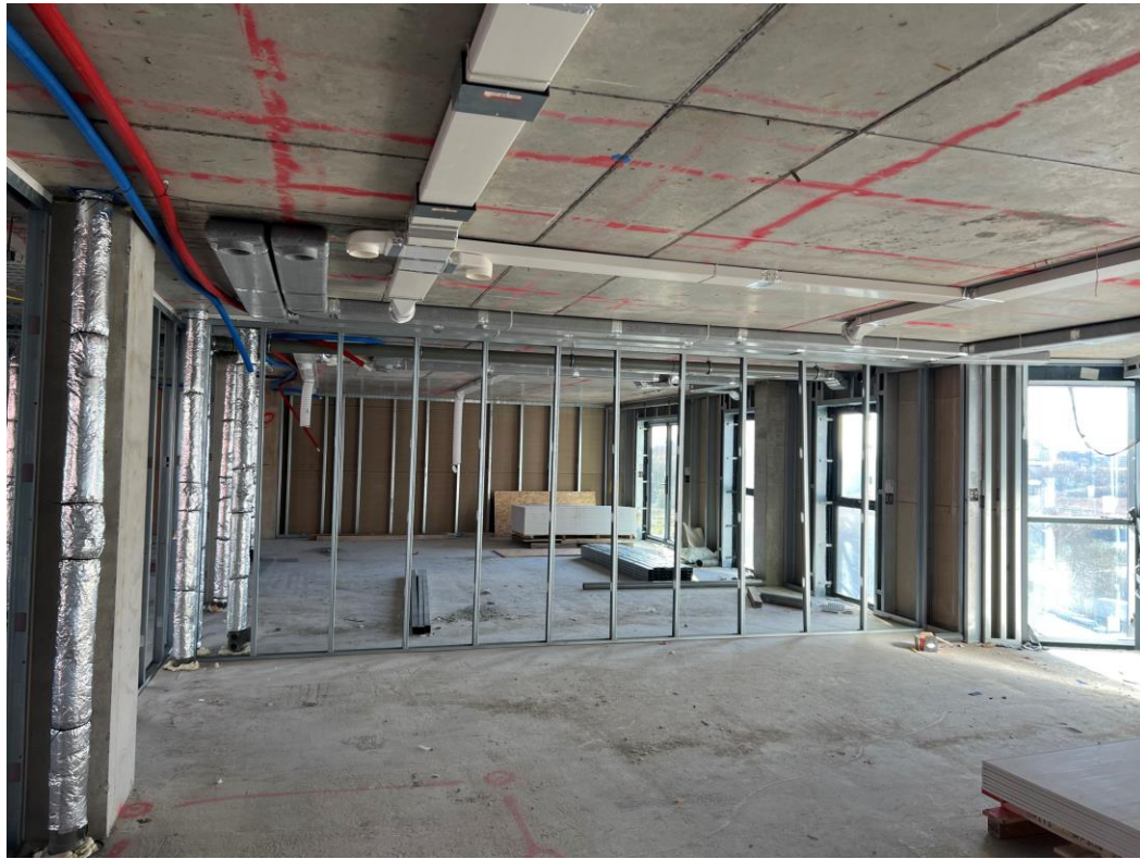
Upper floor mechanical services ongoing
