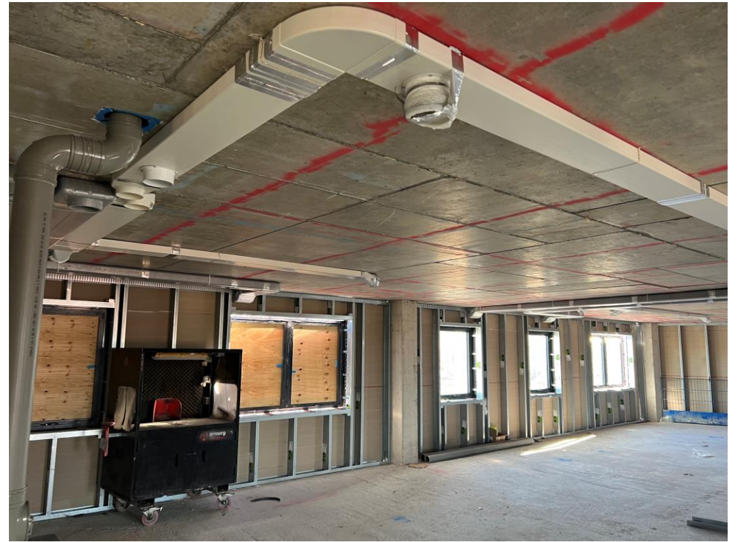
Upper level 1 st fix mechanical ducting & water
