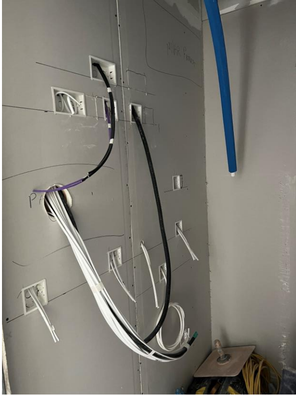
Apartment 1 st fix electrical
