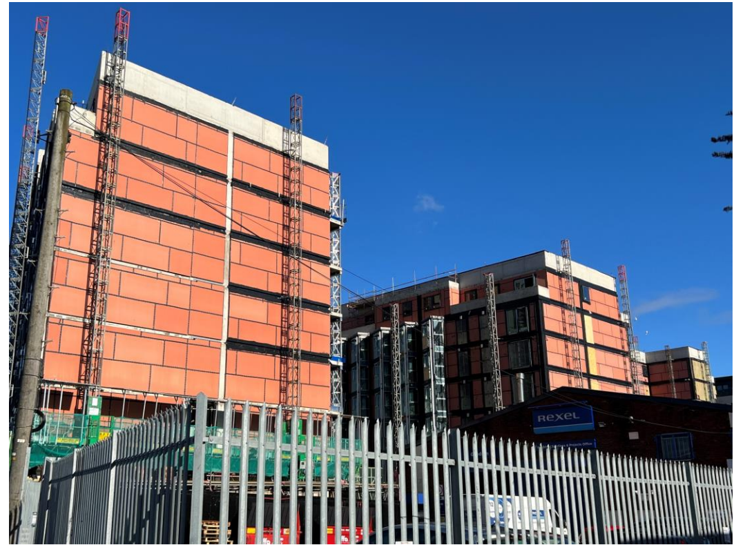
Worrall Street site view
