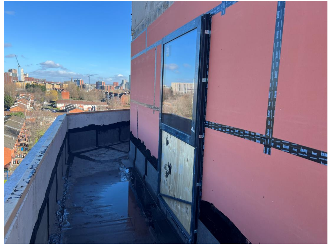
Block A terrace roof covering
