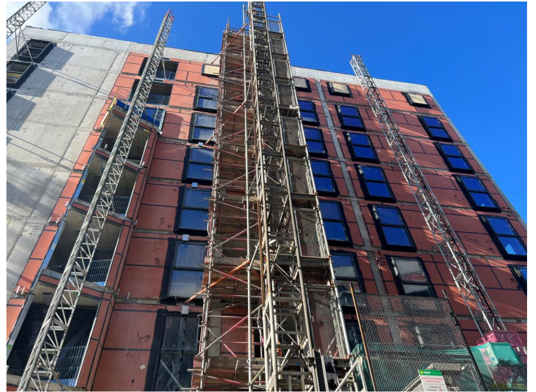
Block A weatherboarding & windows installed
