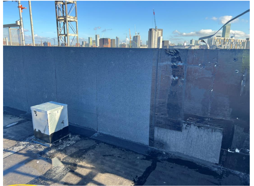
Block A roof covering
