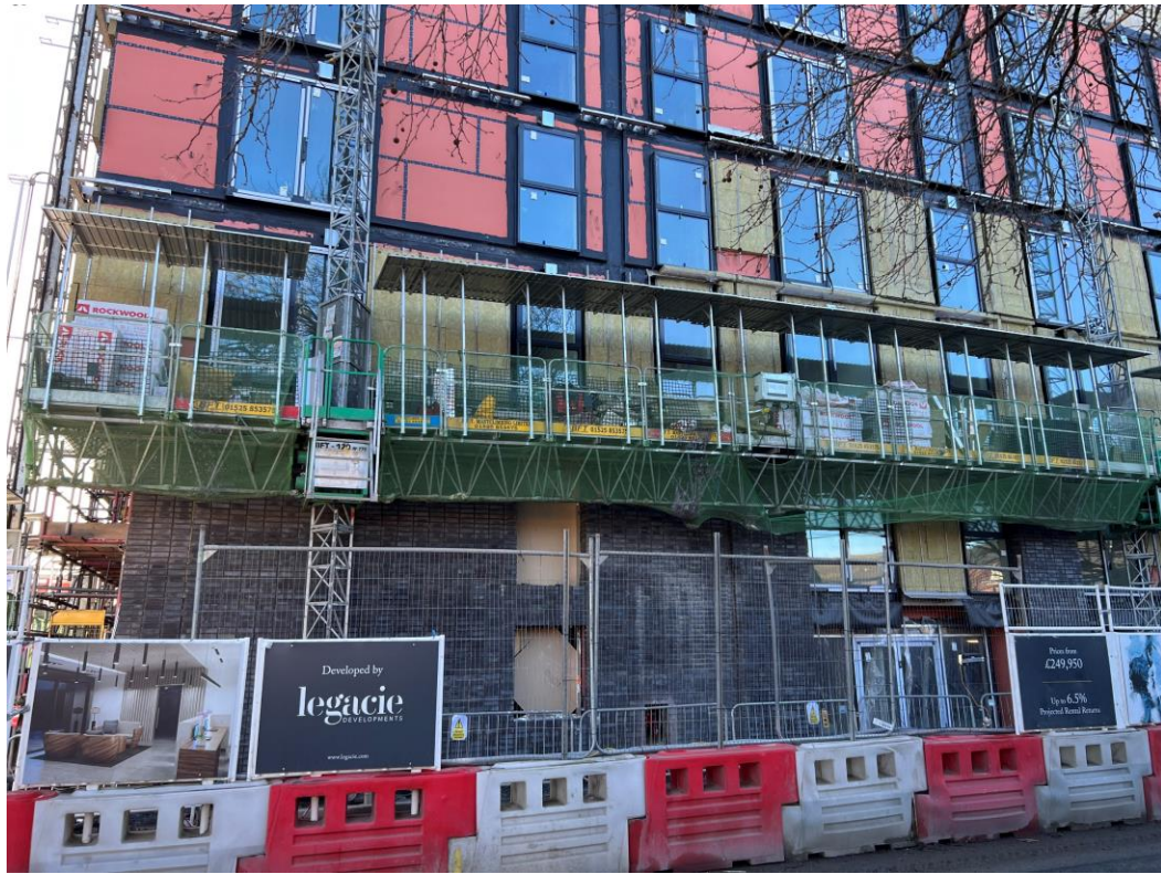
Ordsall Lane site view
