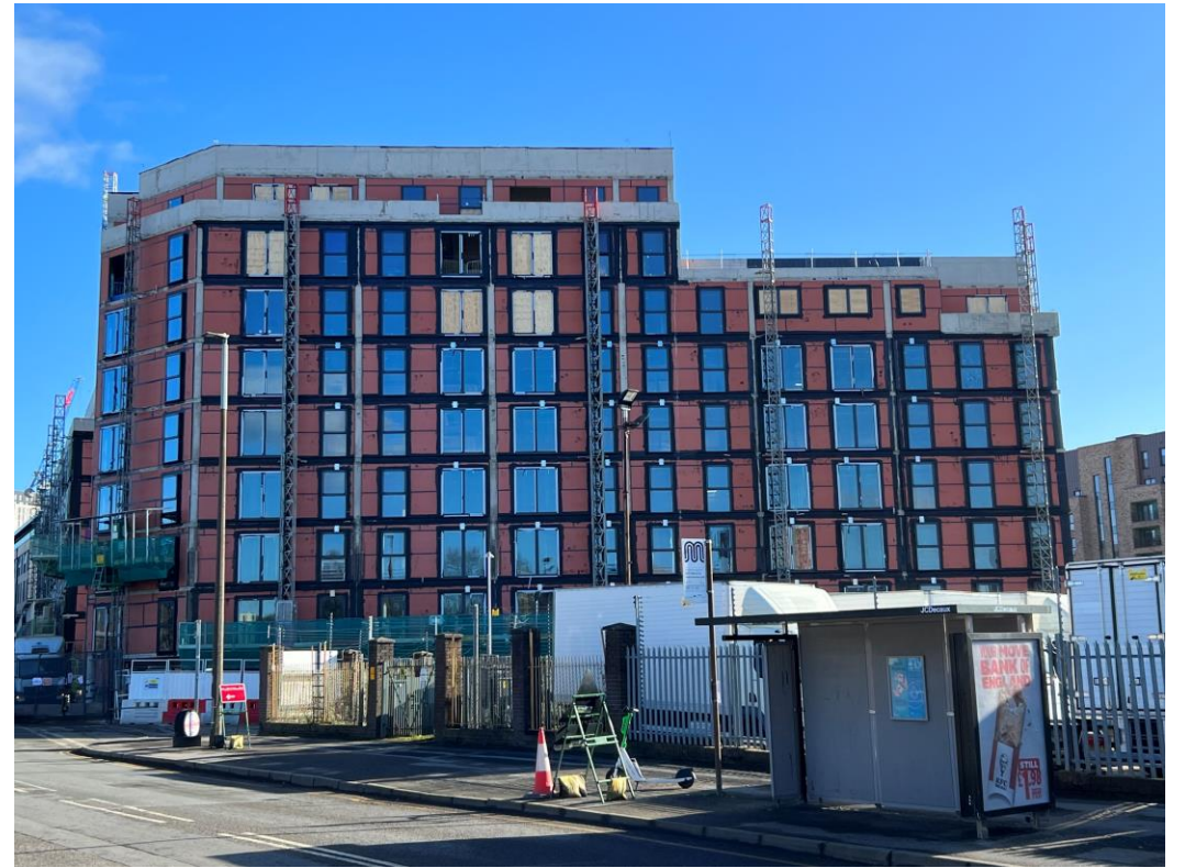
Ordsall Lane site view
