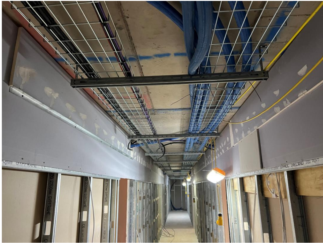
Water main services installation
