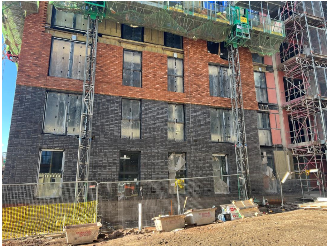
Block B facing brickwork
