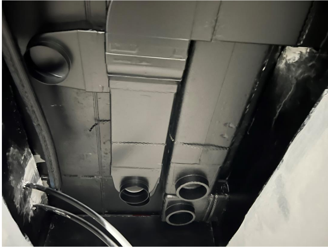
Apartment 2 nd fix mechanical
