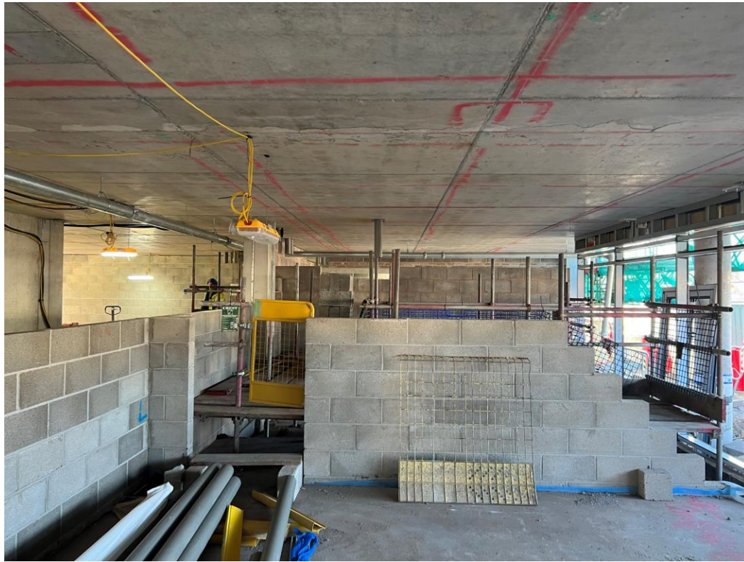
Ground level walls formed
