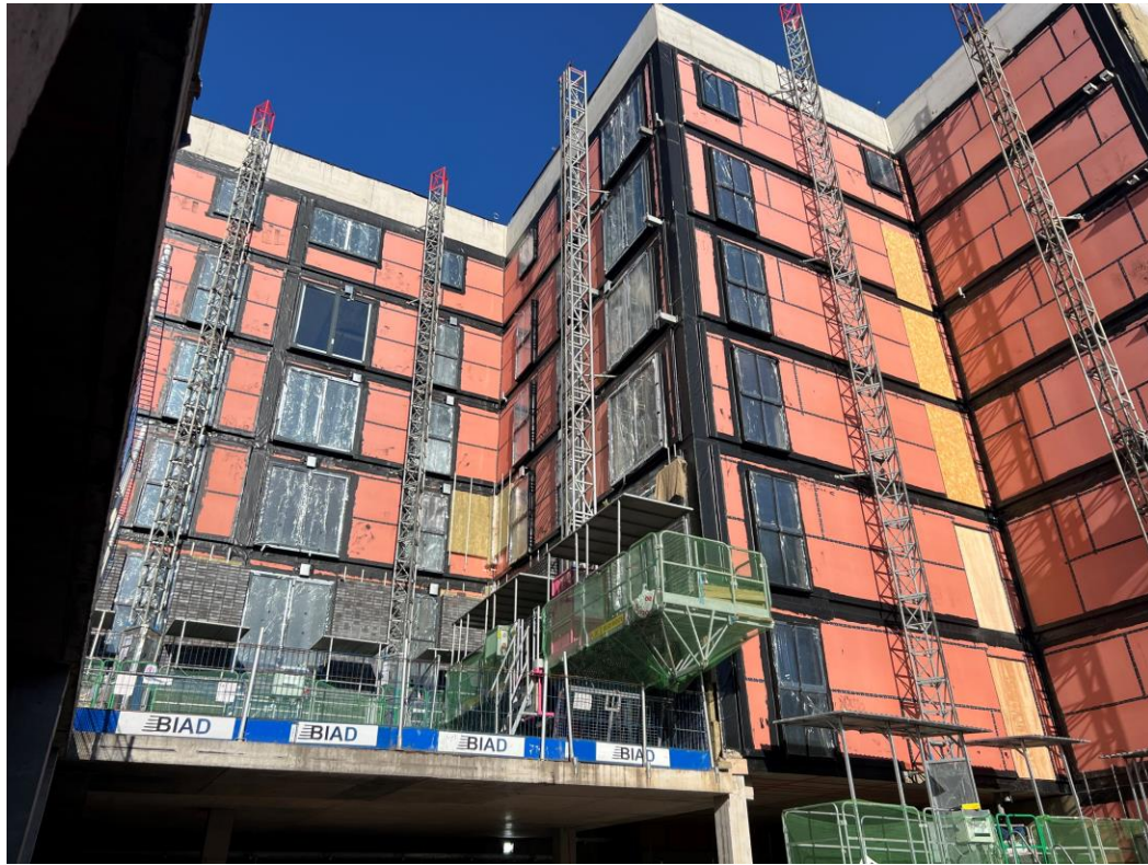
Block B weatherboarding & windows installed
