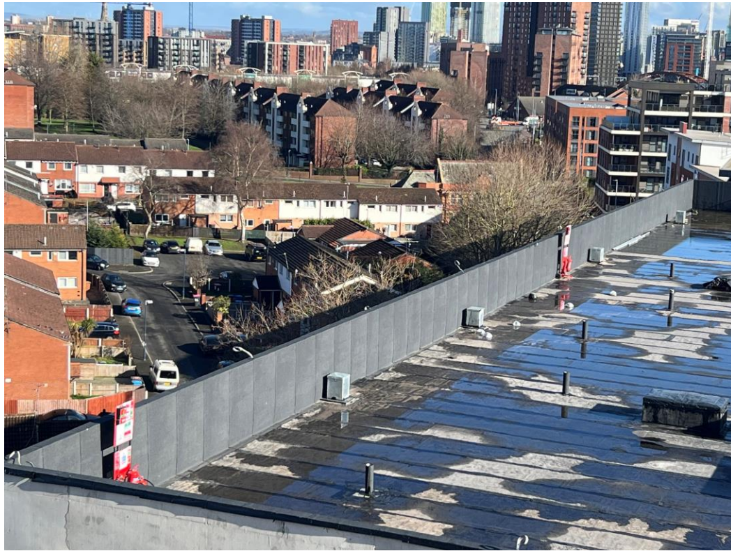
Block B roof covering
