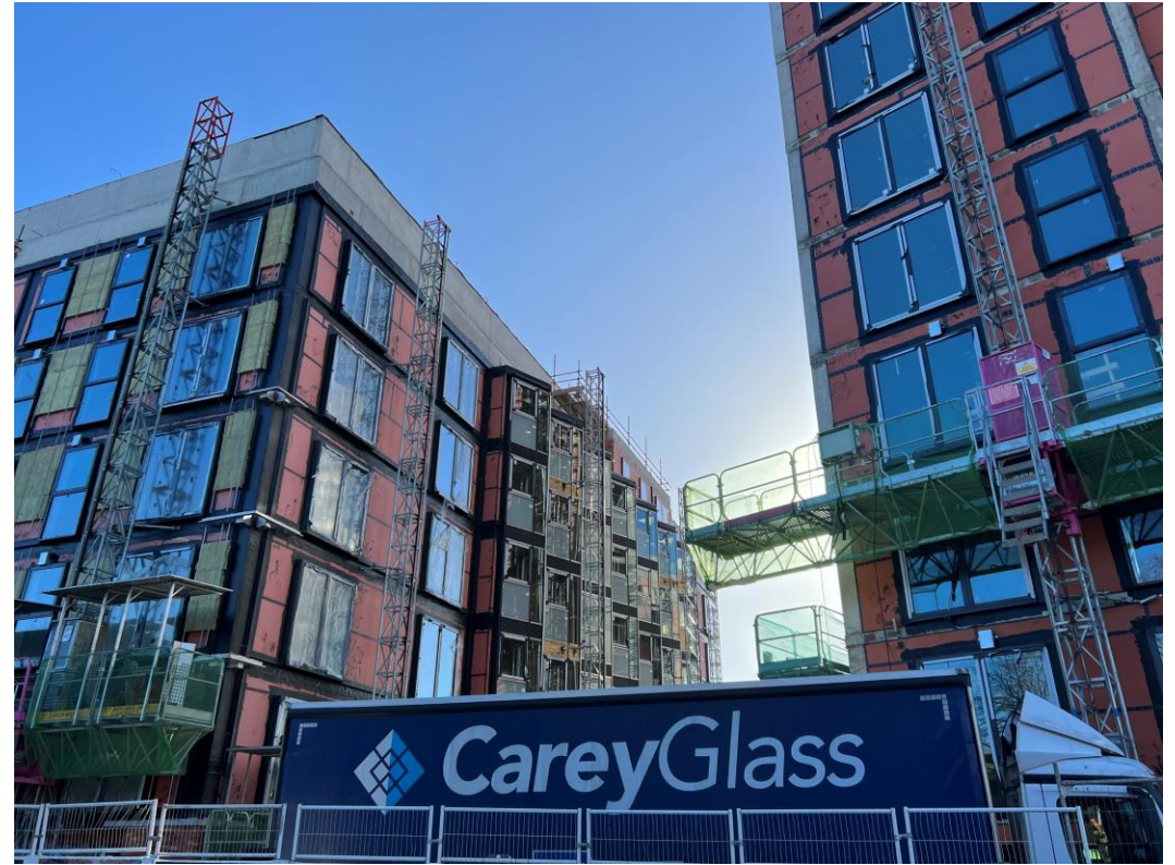
Ordsall Lane site view
