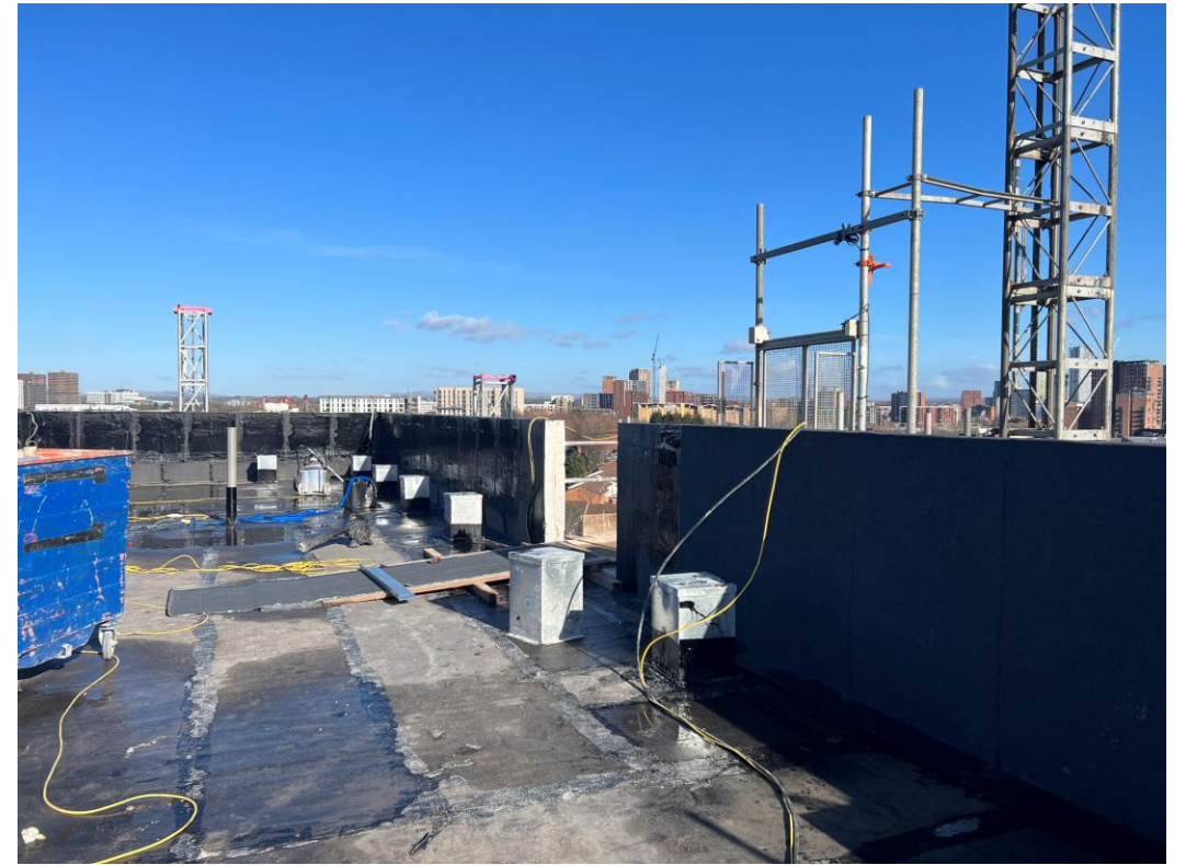
Block A roof covering
