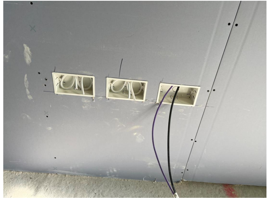
Apartment 1 st fix electrical
