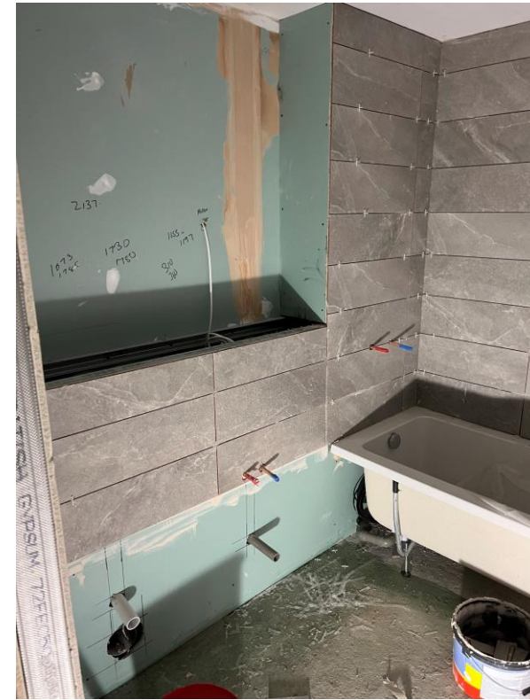
Wall and floor tiling commenced
