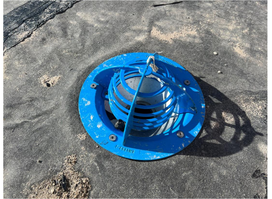
Block A rainwater outlet
