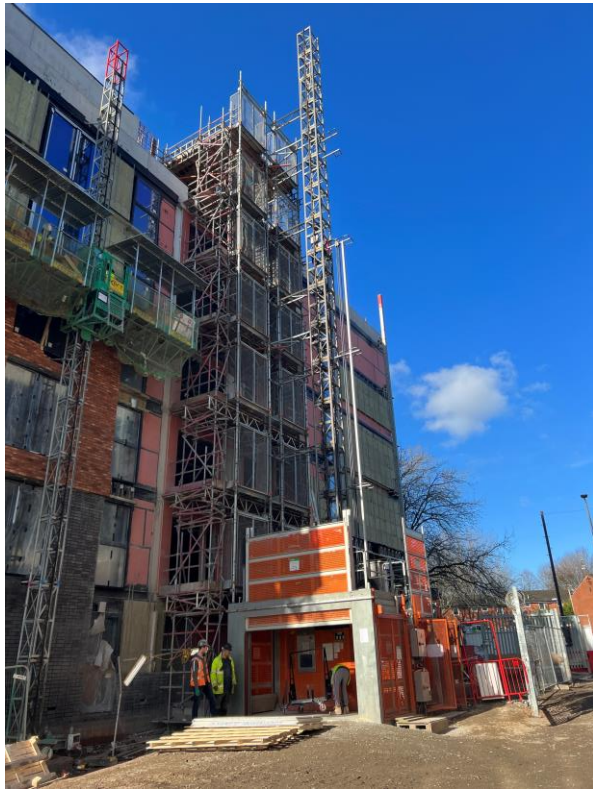
Block B facing brickwork
