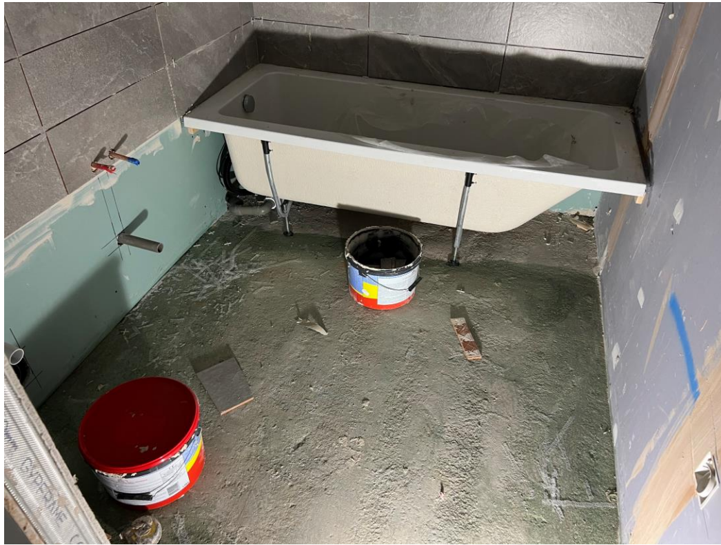
Wall and floor tiling commenced
