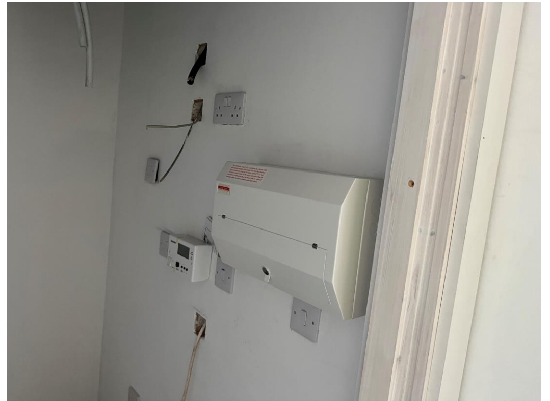
2 nd fix electrical
