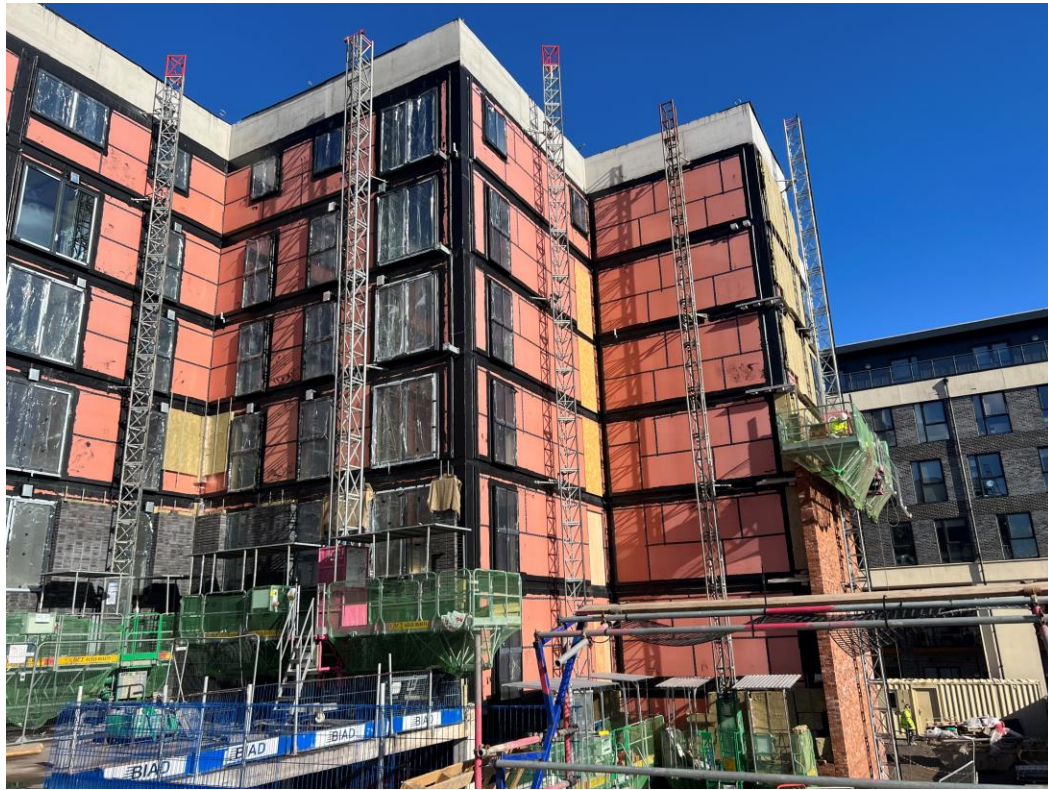
Block B Podium facing brickwork
