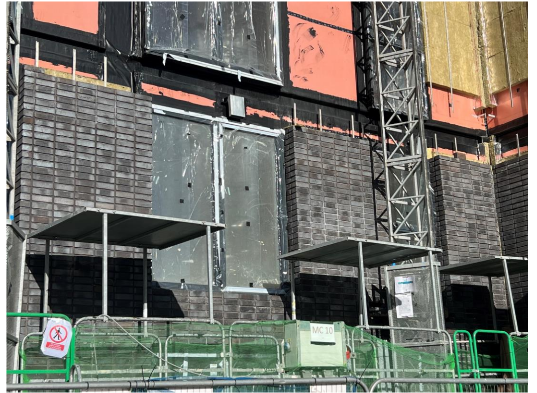
Block B Podium facing brickwork
