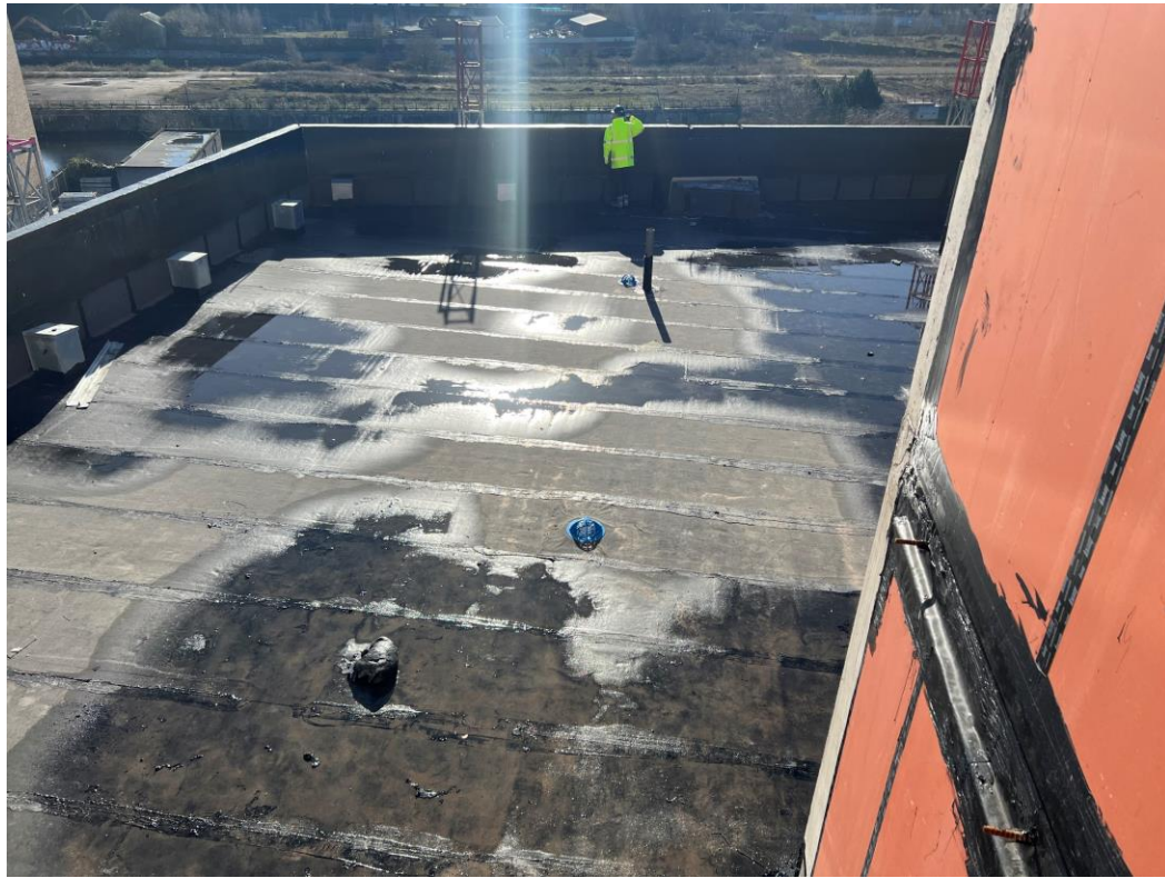
Block A terrace roof covering
