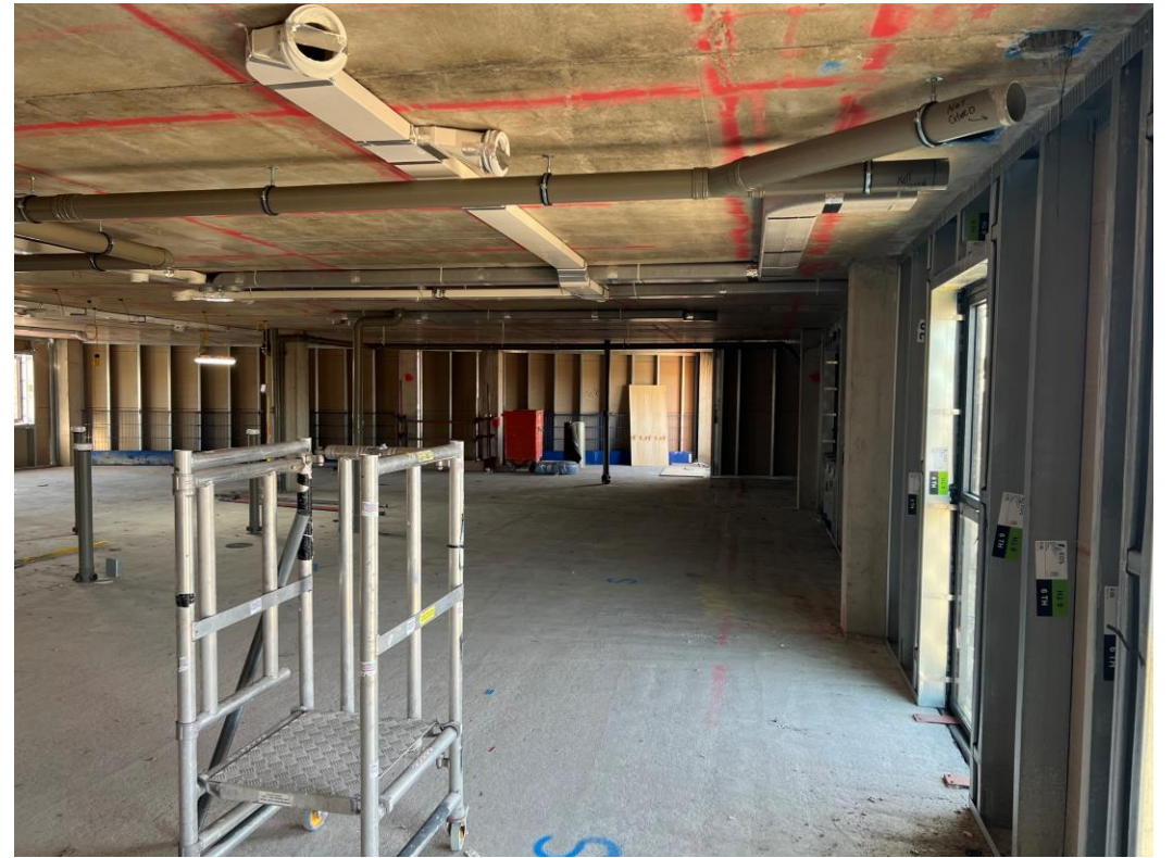
Upper level 1 st fix mechanical ducting & water
