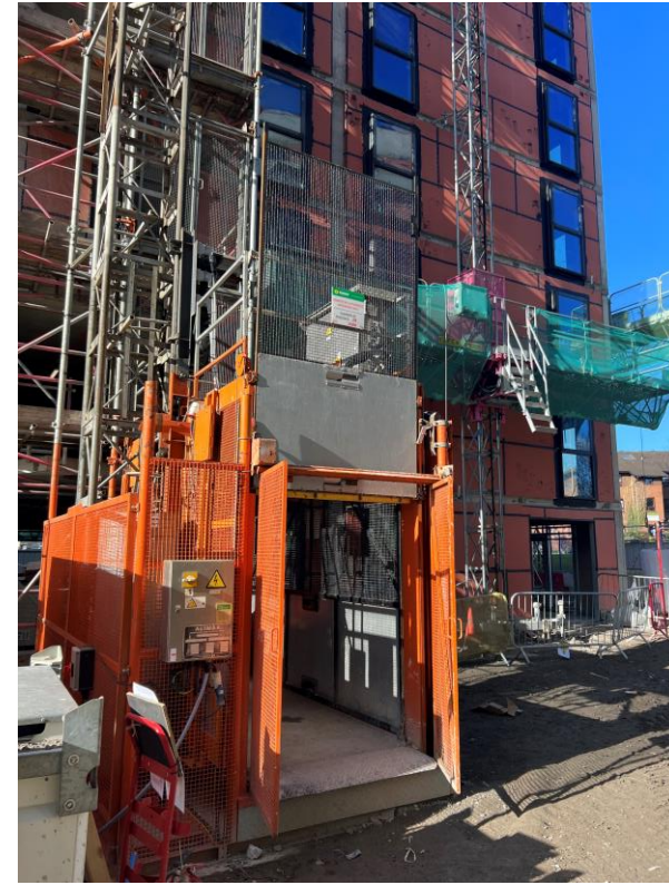
Block A weatherboarding & windows installed
