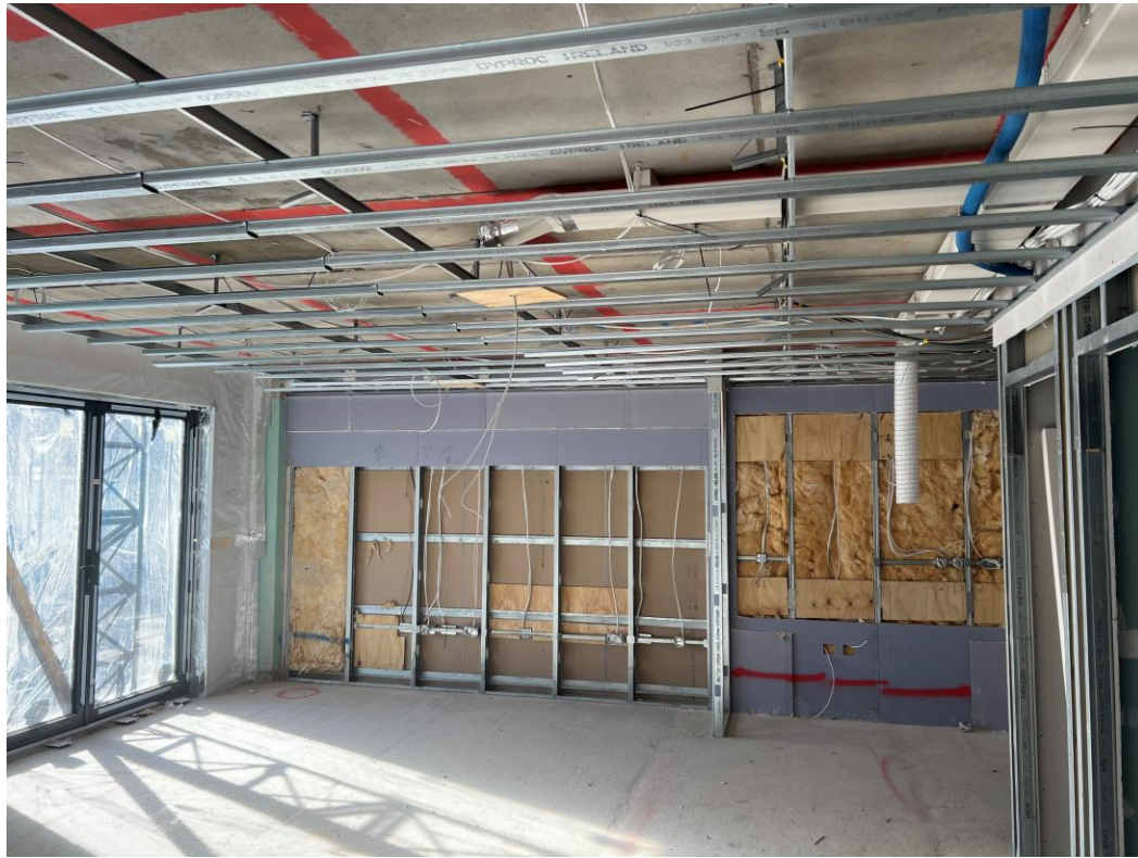
Upper floor Apartment partitions ongoing
