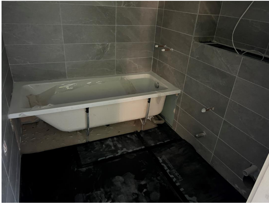
Wall and floor tiling commenced
