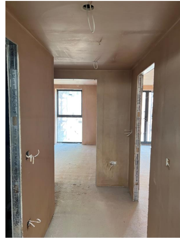
Upper level Apartment plaster skim ceiling and walls
