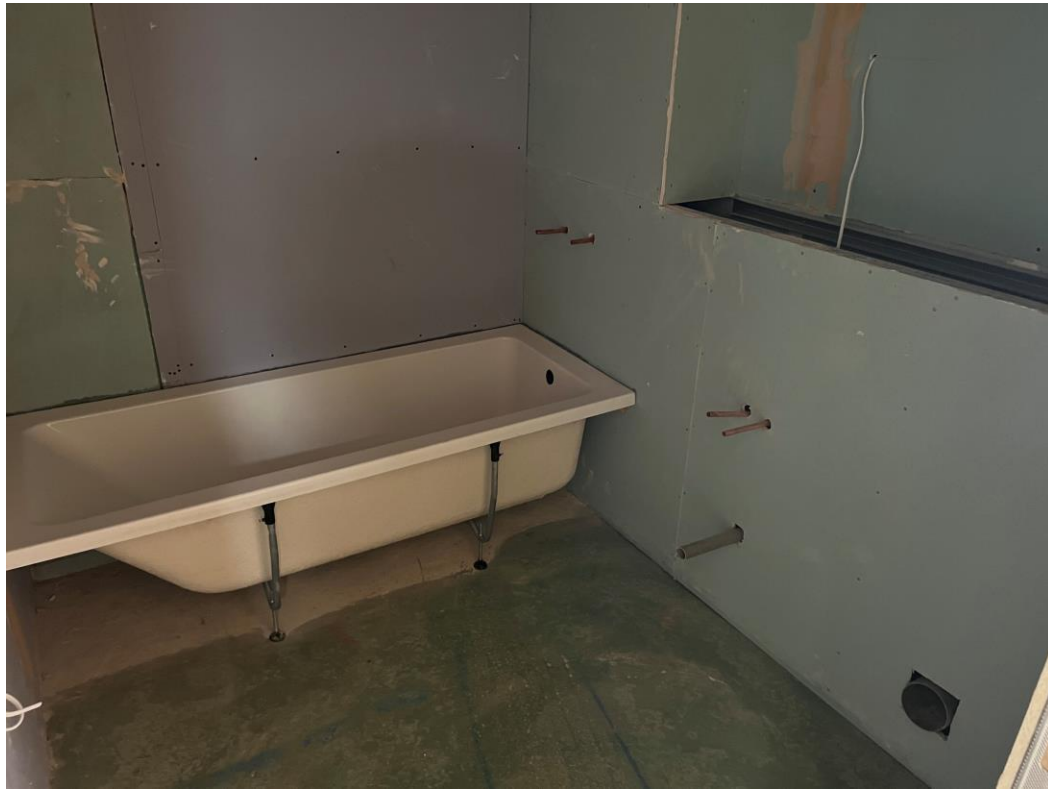
Sanitary installation commenced
