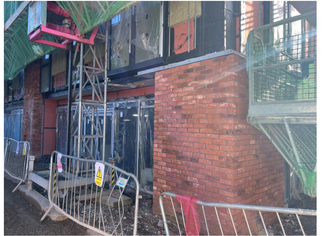
Block B weatherboarding & windows installed
