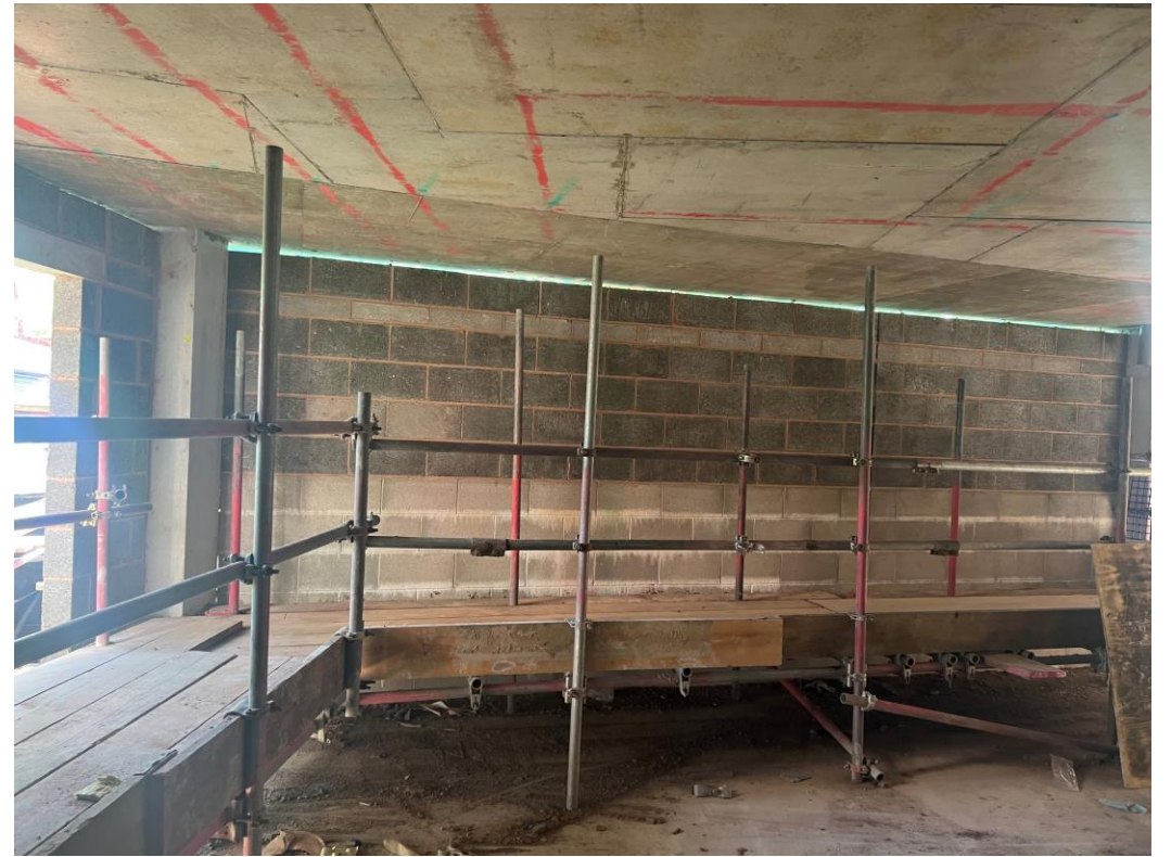
Ground level walls formed
