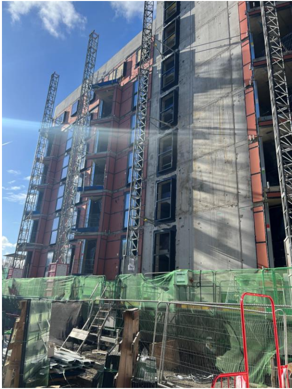
Block A weatherboarding & windows installed
