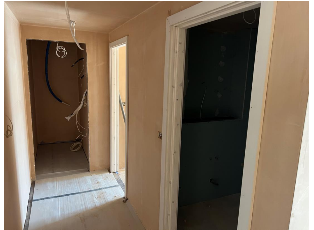
Doorframes, skirting and architrave
