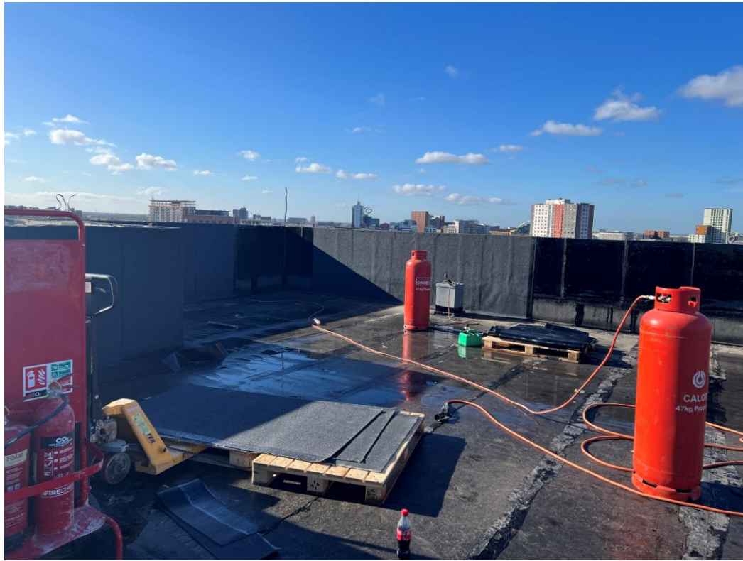
Block A roof covering
