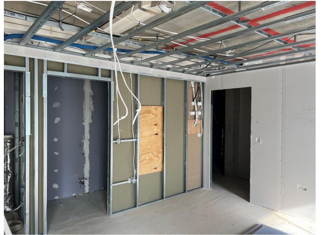
Upper floor Apartment partitions ongoing
