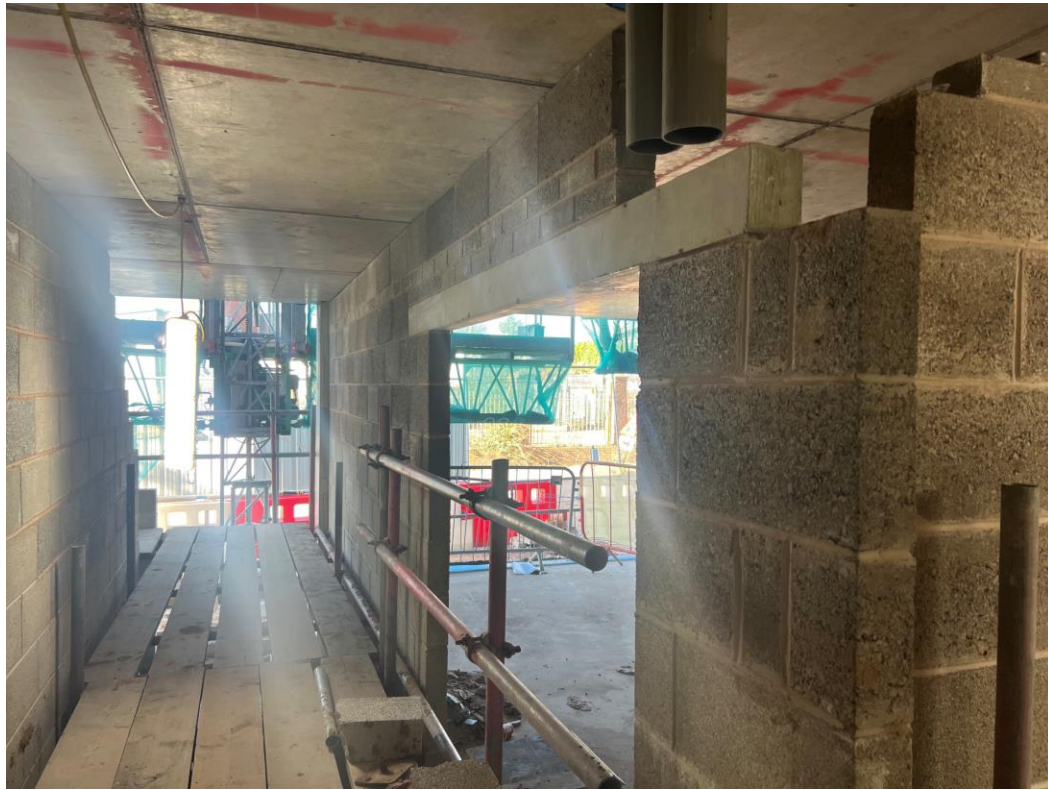
Ground level walls formed
