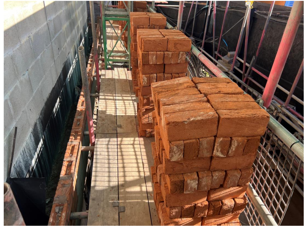
Block A facing brickwork
