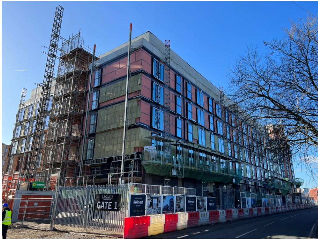
Ordsall Lane site view
