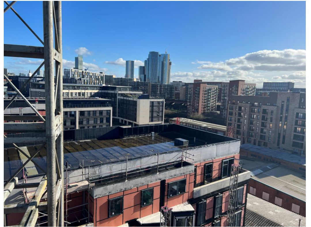
Block B roof covering
