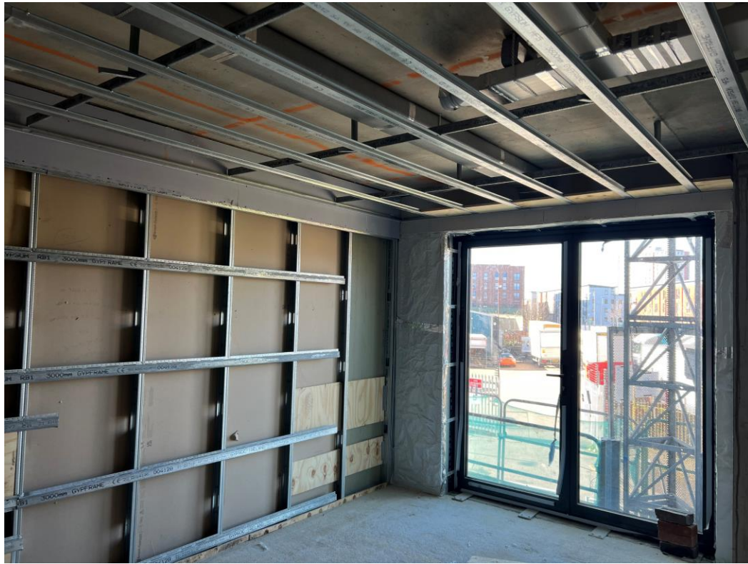
1 st Floor partition walls and ceiling
