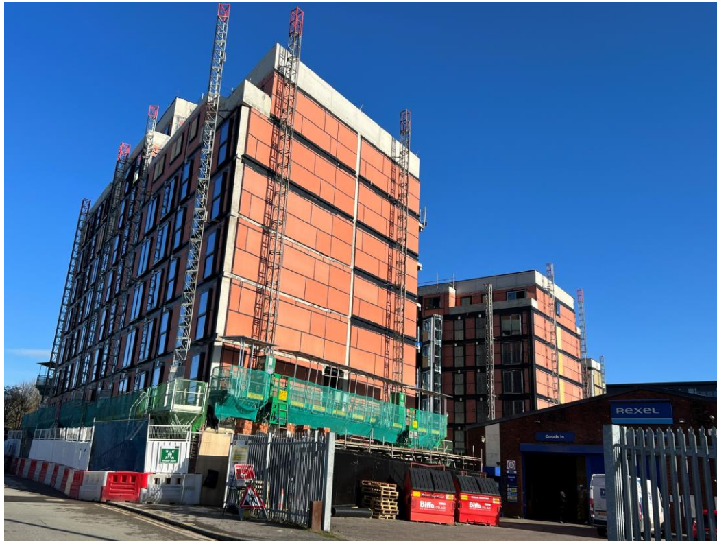
Worrall Street site view
