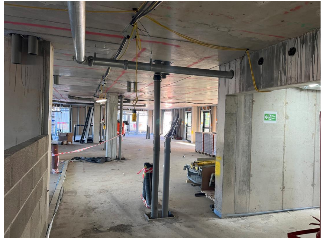
Ground level walls formed
