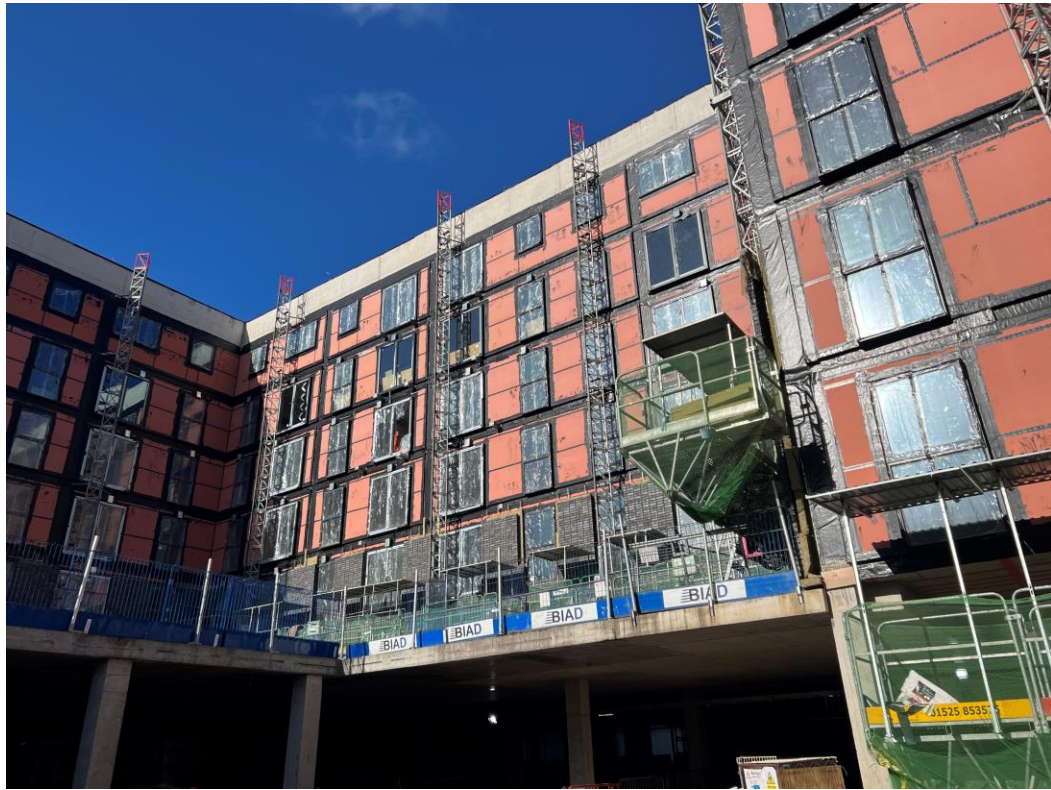
Block B facing brickwork
