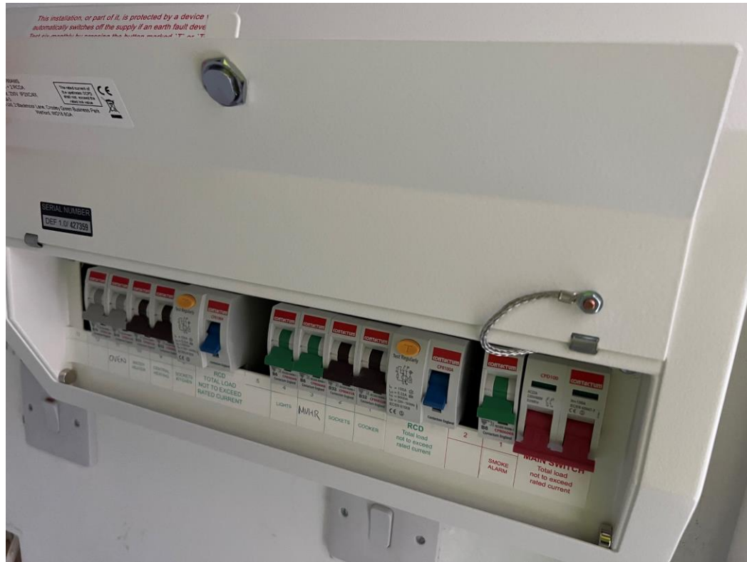
2 nd fix electrical
