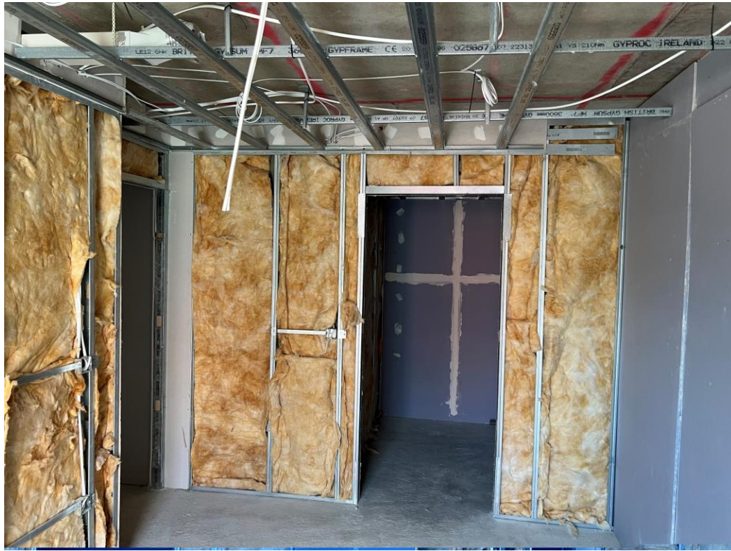
Upper floor Apartment partitions ongoing
