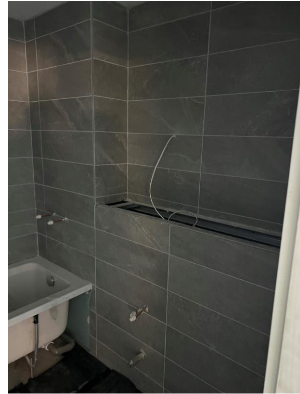
Wall and floor tiling commenced
