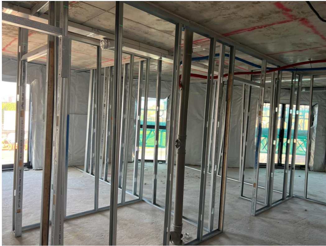
2 nd Floor partition walls
