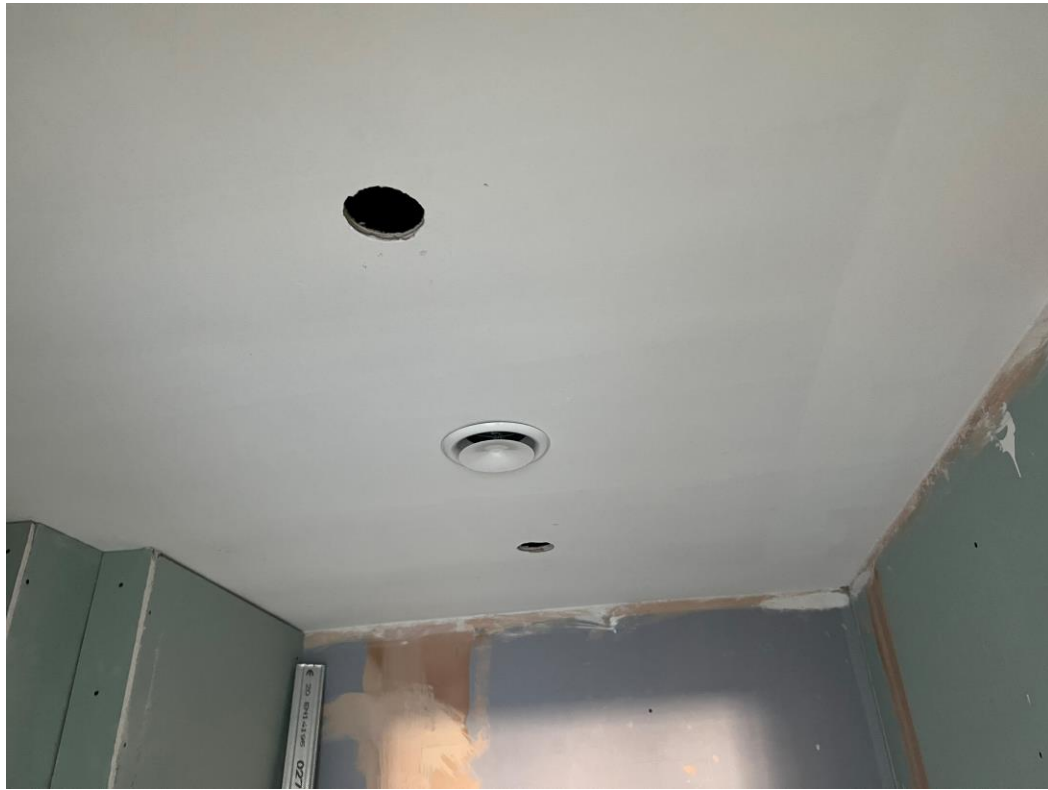
Apartment 2 nd fix mechanical
