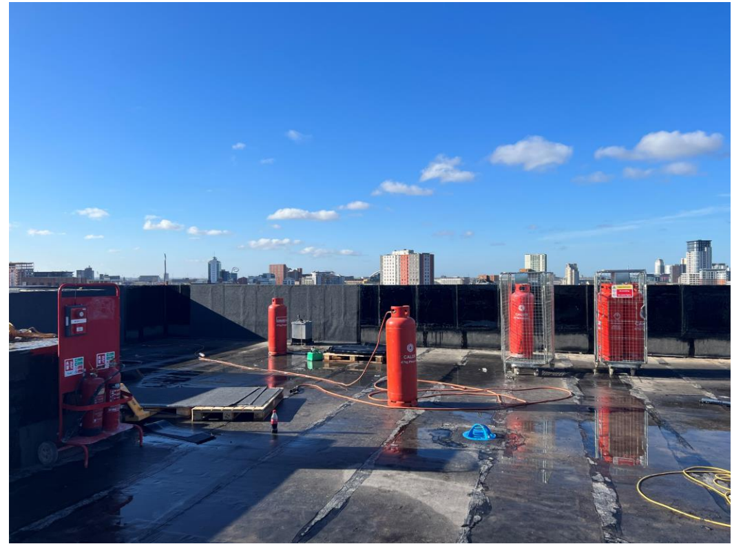
Block A roof covering
