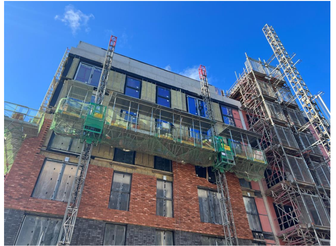
Block B facing brickwork
