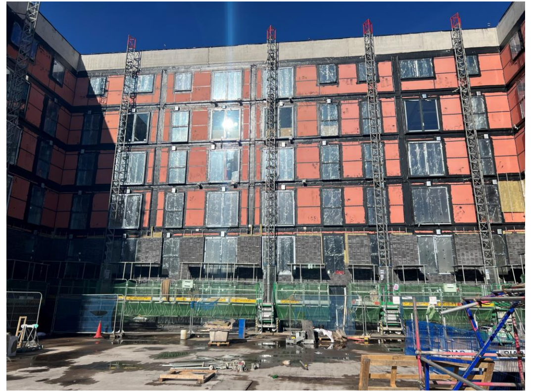
Block B Podium facing brickwork
