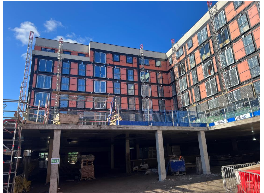
Block B facing brickwork
