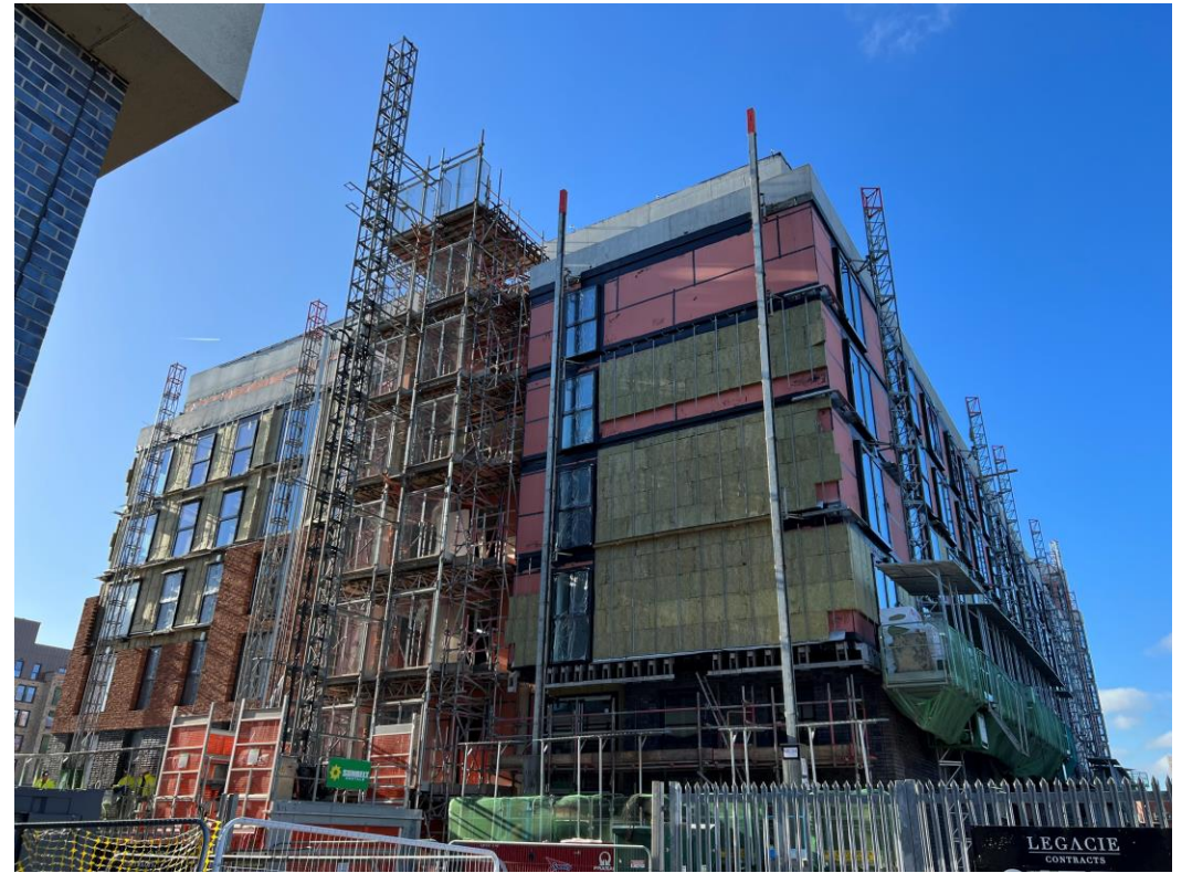
Ordsall Lane site view
