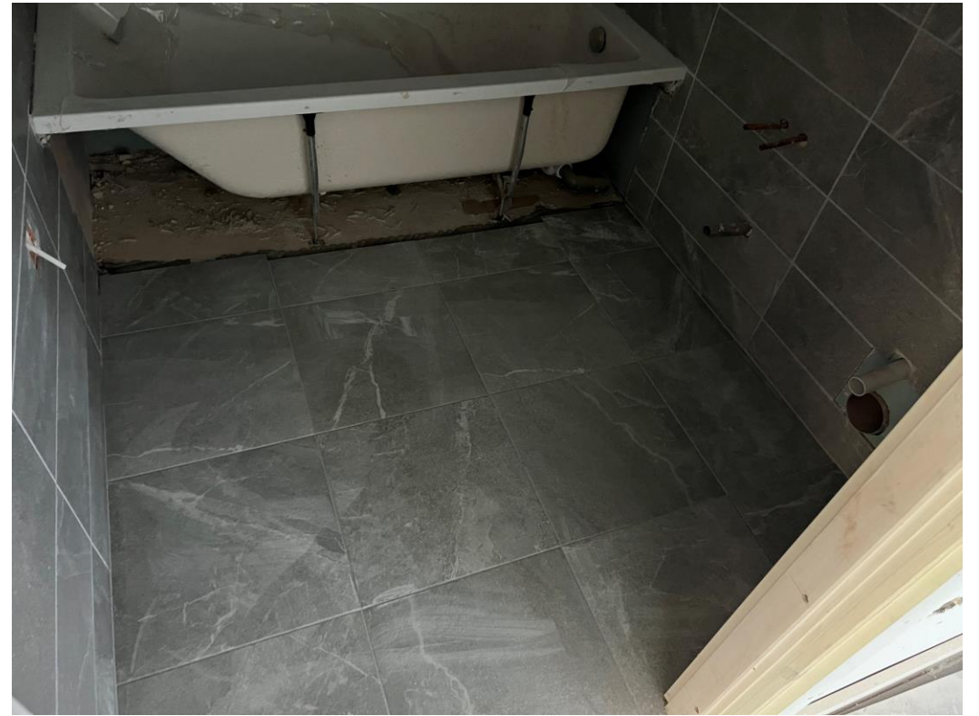
Wall and floor tiling commenced
