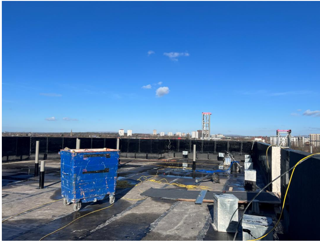
Block A roof covering
