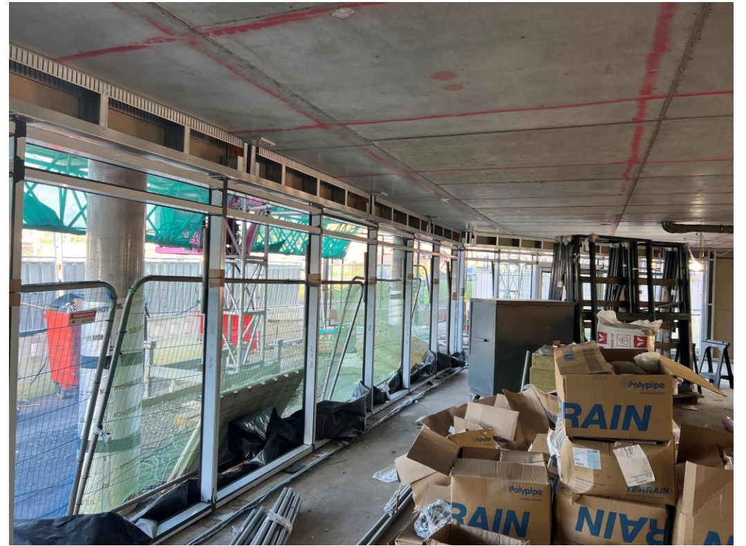
Curtain wall framing installed
