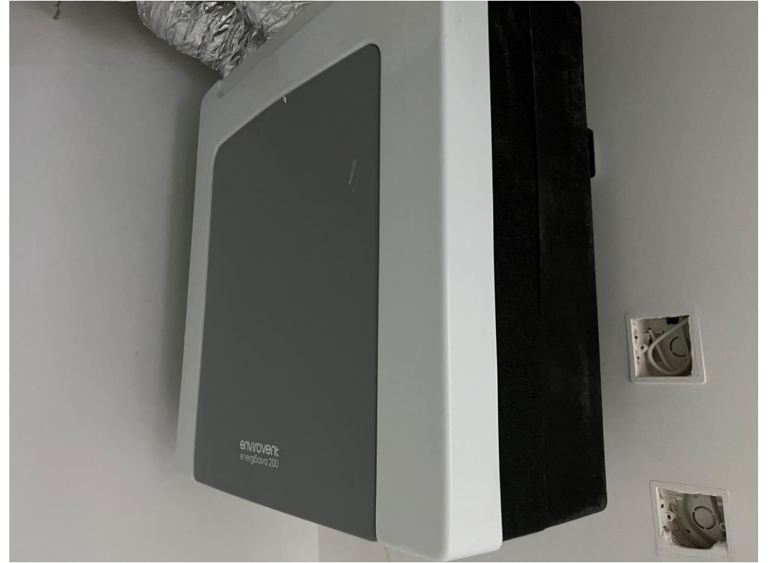
Apartment 2 nd fix mechanical
