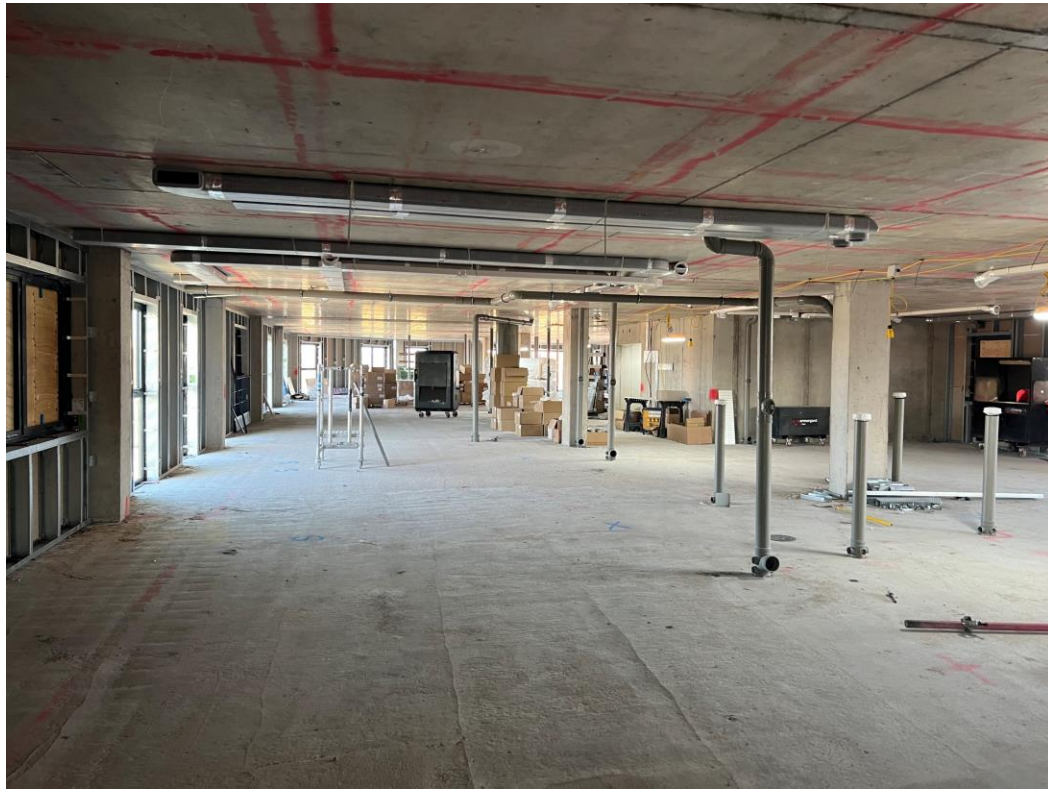
Upper level 1 st fix mechanical ducting & water
