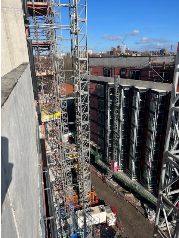
Block B weatherboarding & windows installed
