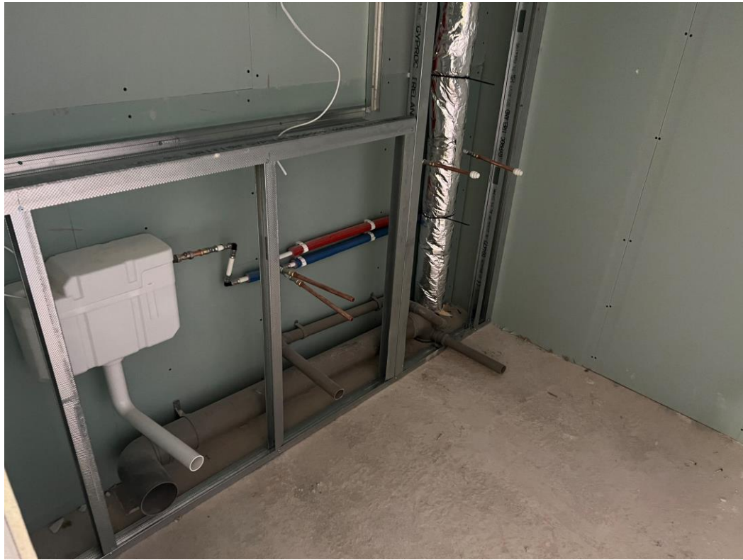
Apartment 1 st fix sanitary
