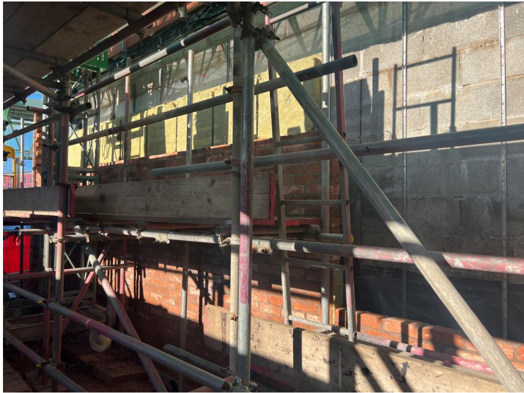
Block A facing brickwork
