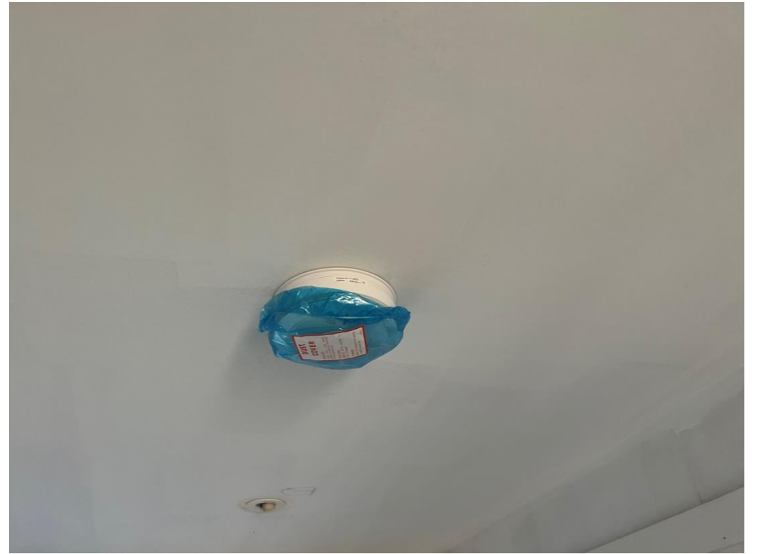
2 nd fix electrical
