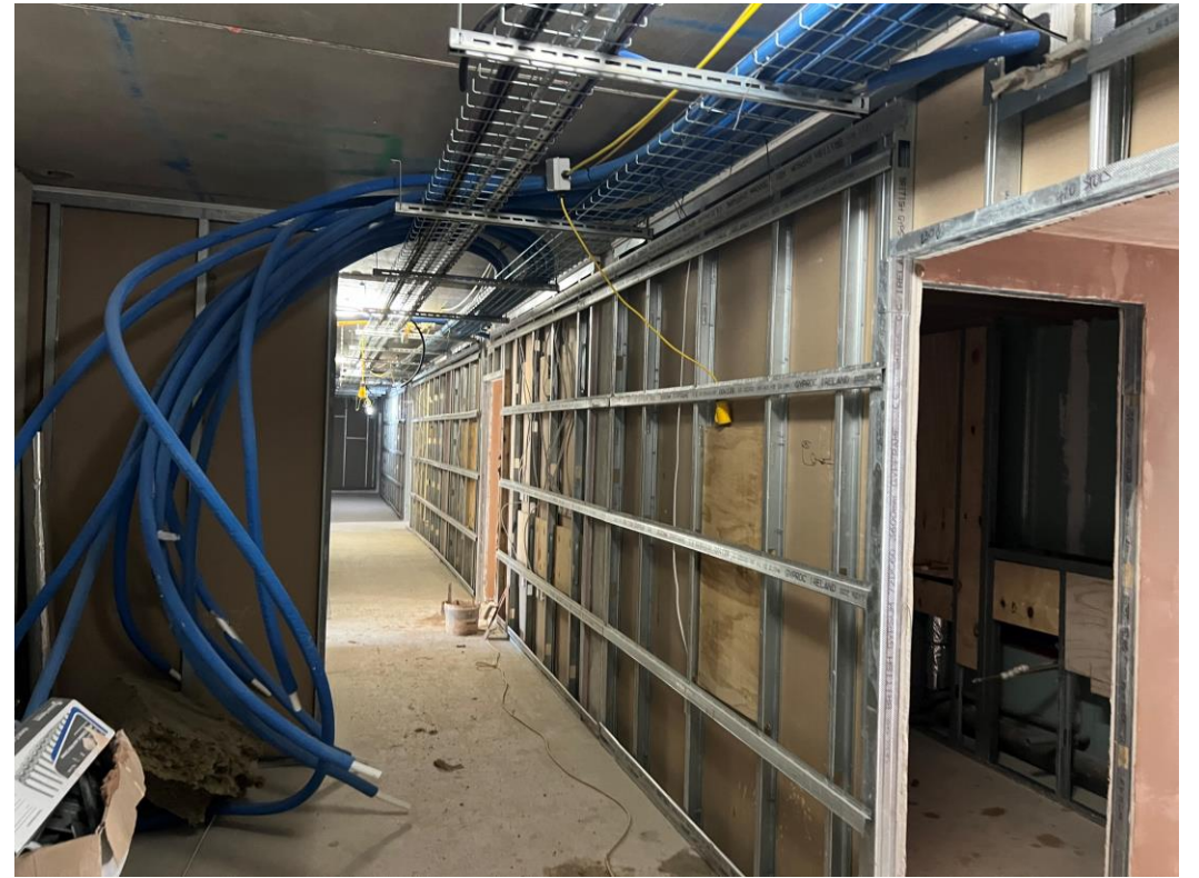
Water main services installation
