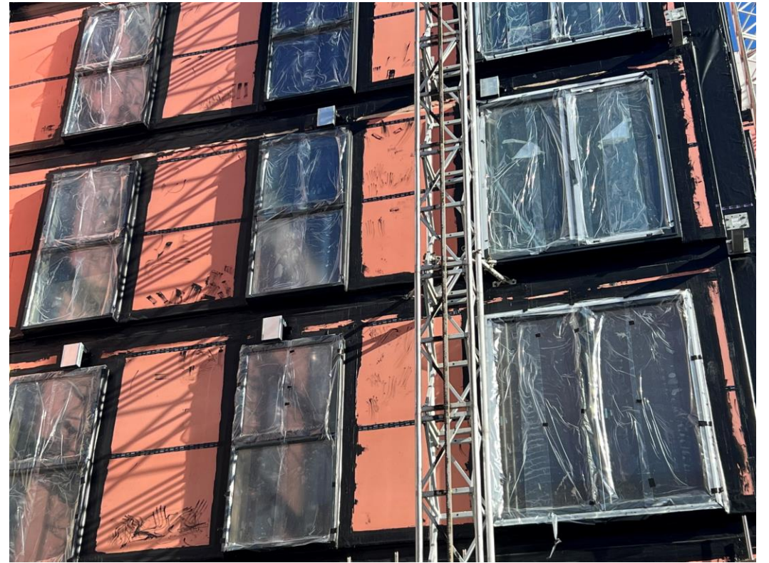
Block B weatherboarding & windows installed
