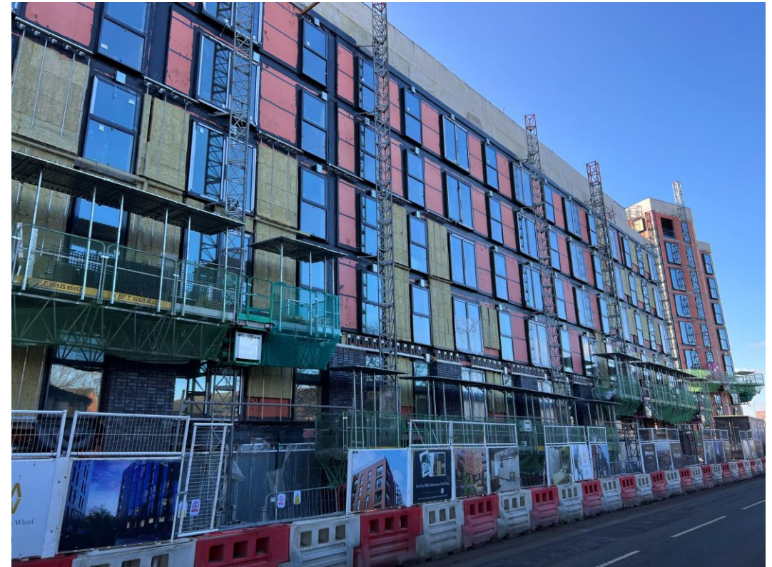
Ordsall Lane site view
