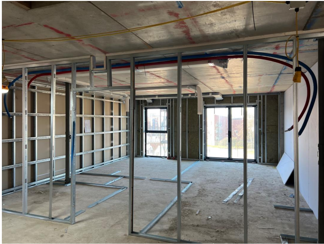
3 rd Floor partition walls
