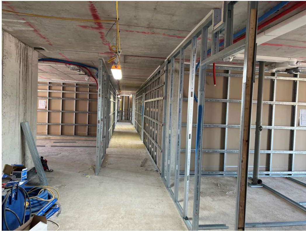
3 rd Floor partition walls
