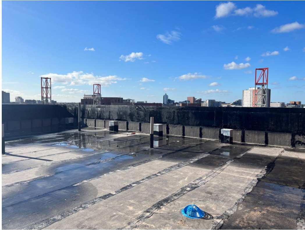
Block A terrace roof covering
