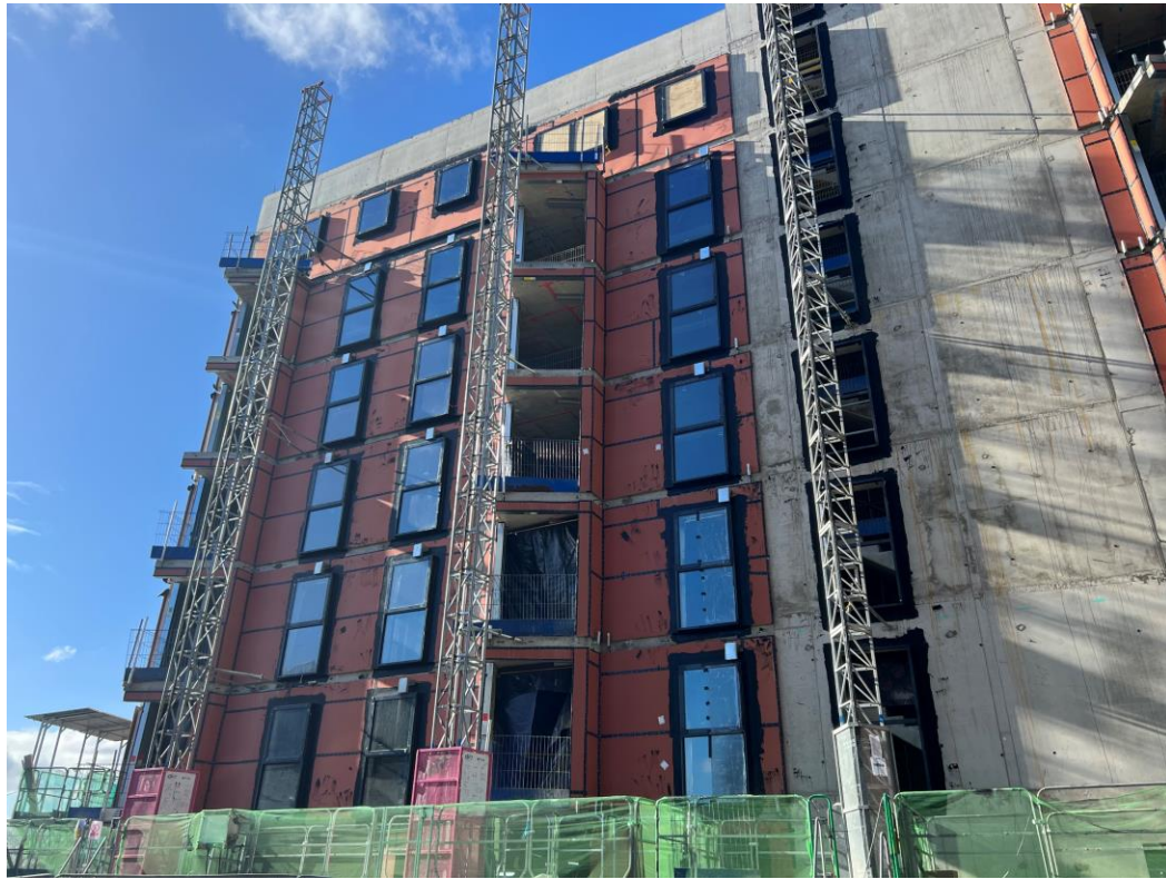
Block A weatherboarding & windows installed
