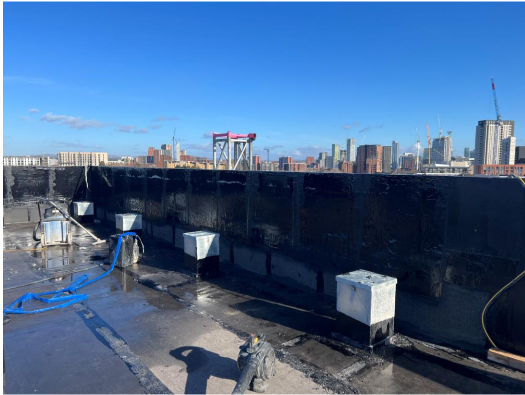
Block A roof covering
