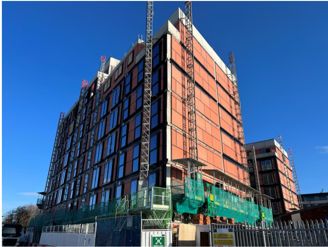
Worrall Street site view
