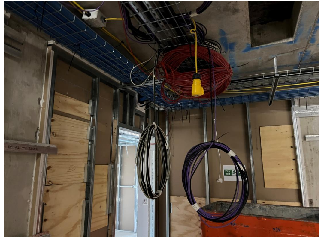
Electrical services installation
