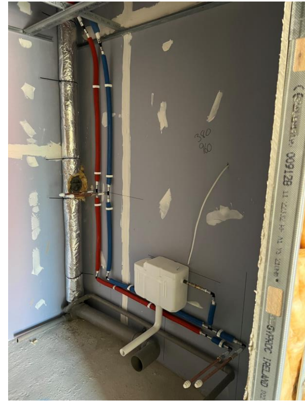
Apartment 1 st fix sanitary
