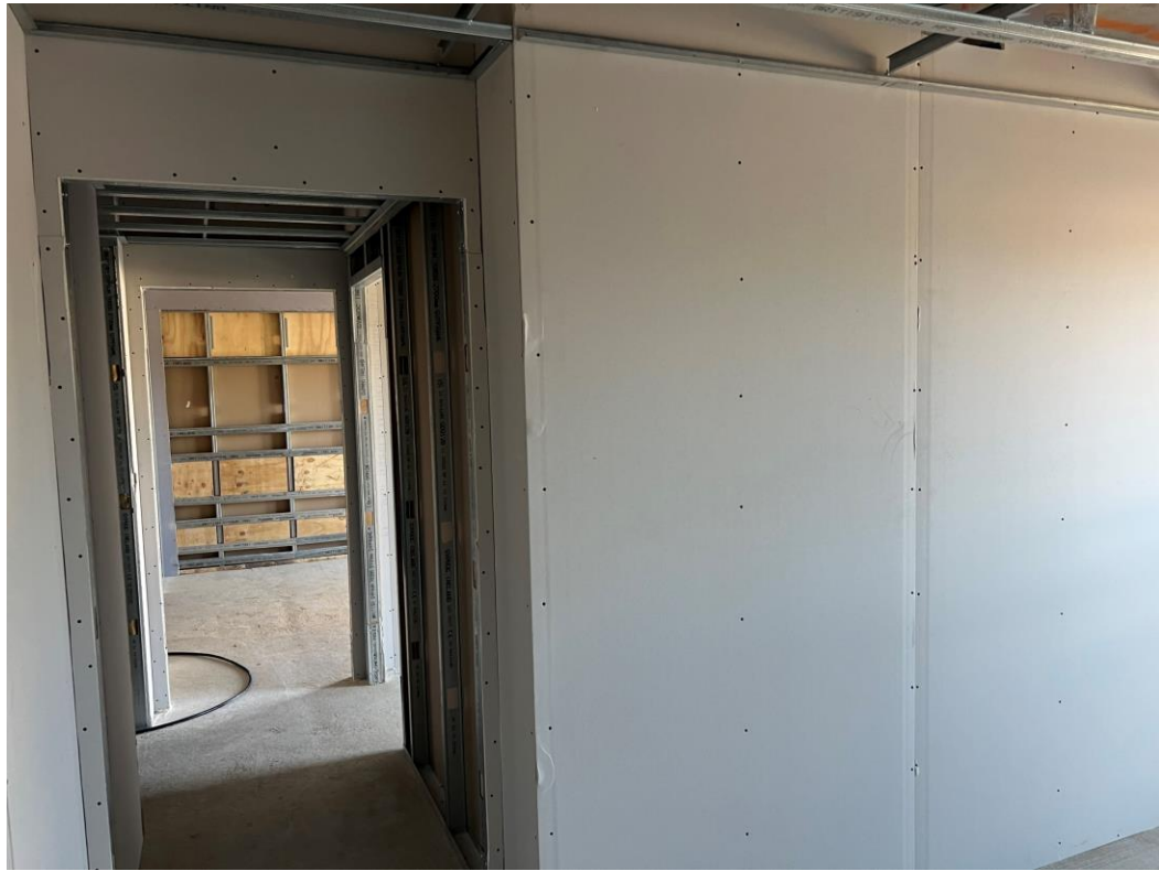
1 st Floor partition walls and ceiling
