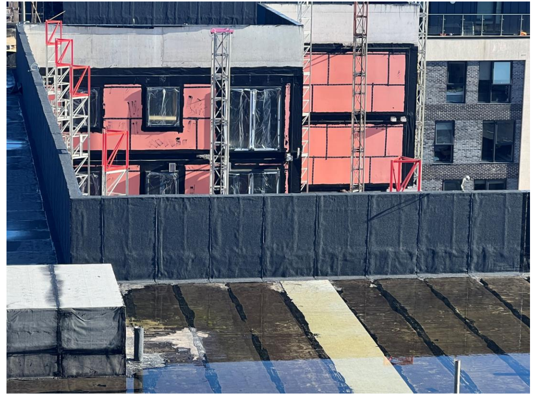
Block B roof covering
