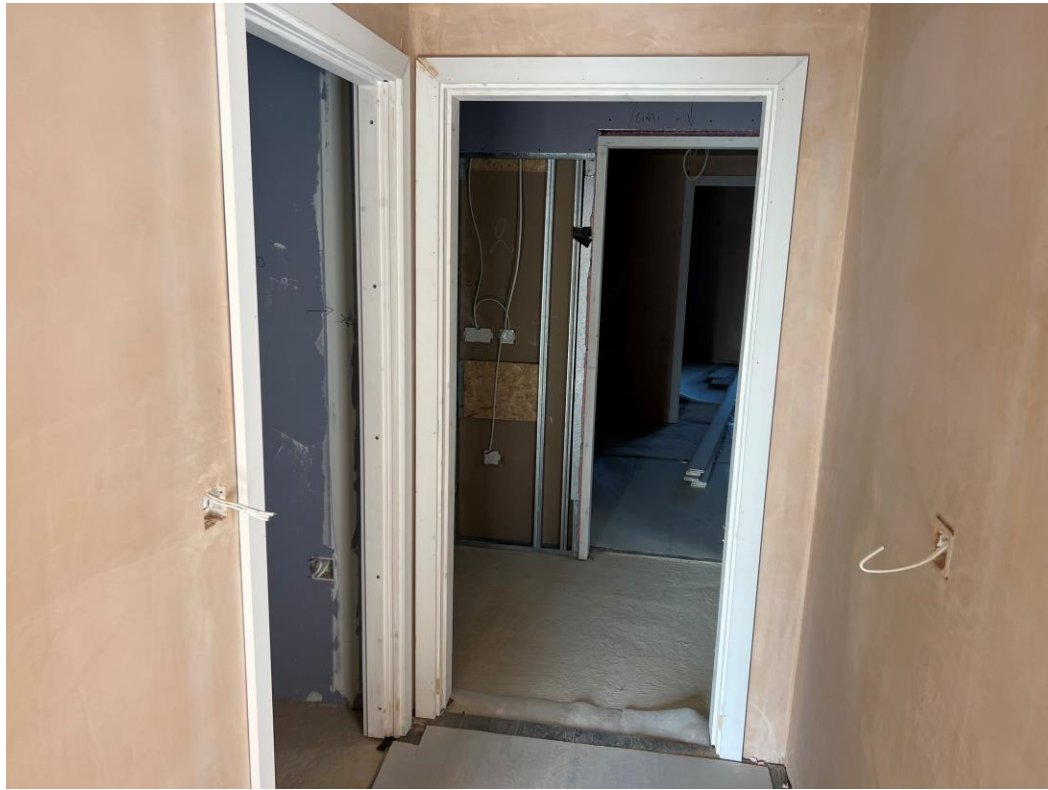
Doorframes, skirting and architrave
