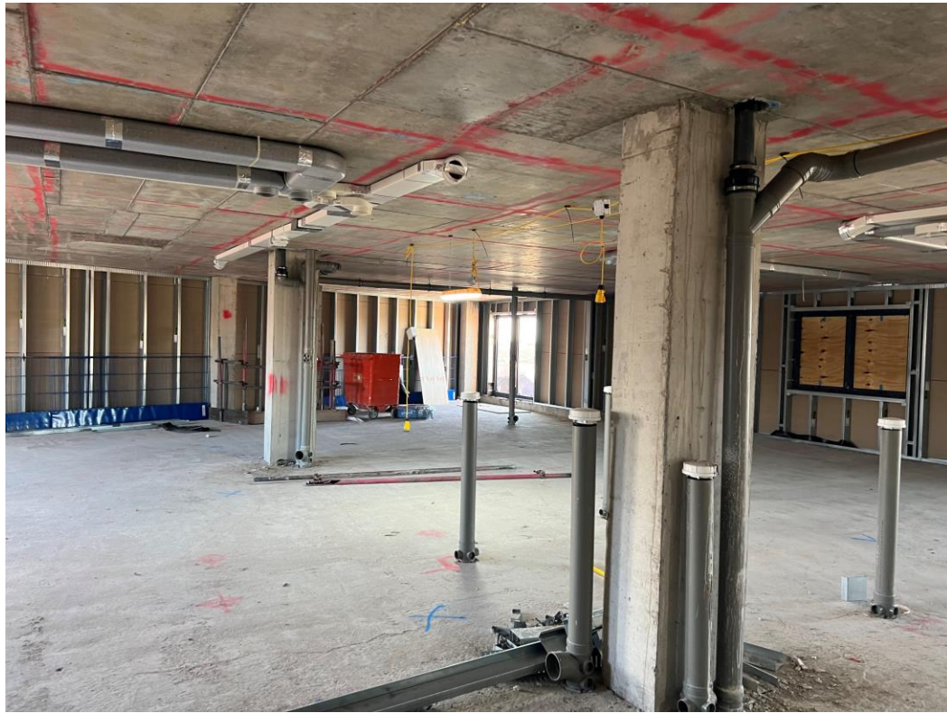
Upper level 1 st fix mechanical ducting & water
