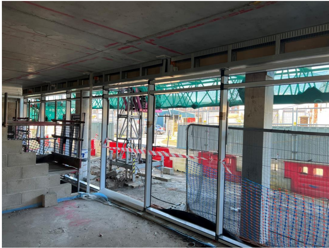
Curtain wall framing installed
