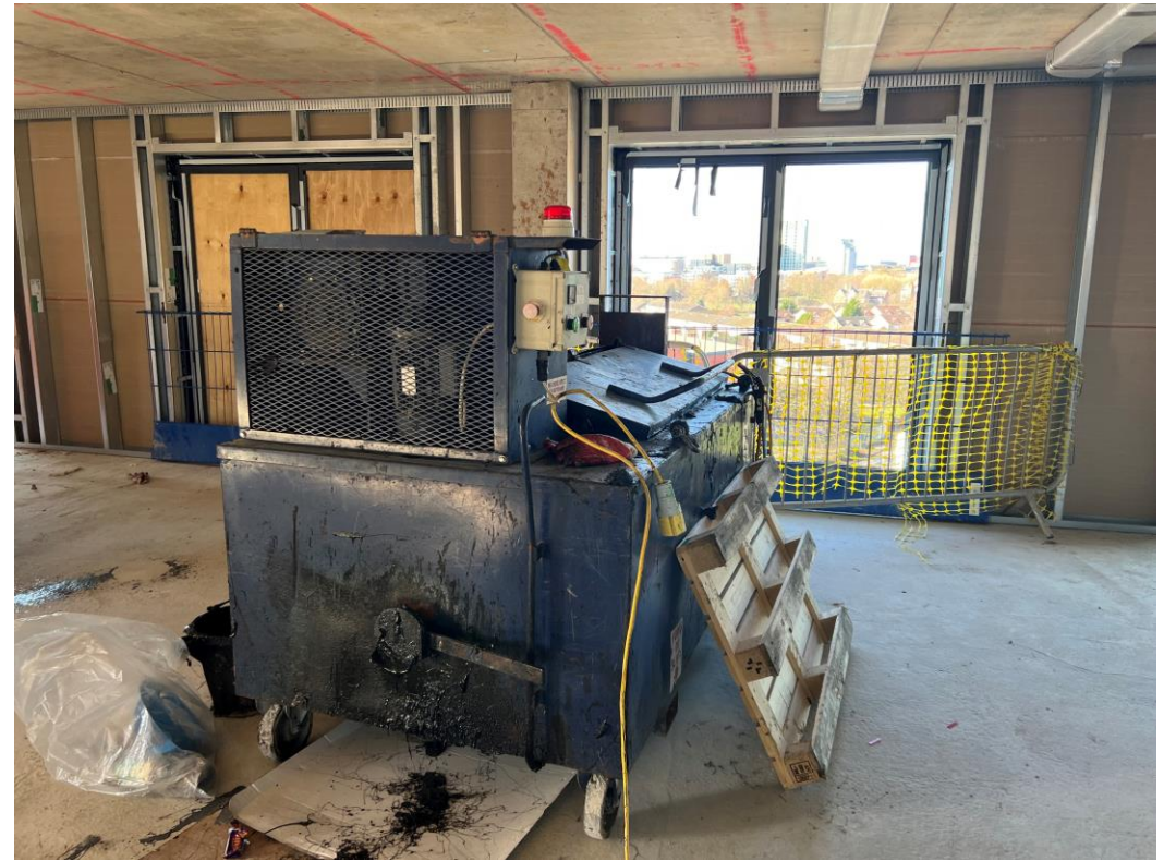
Block A roofing kettle
