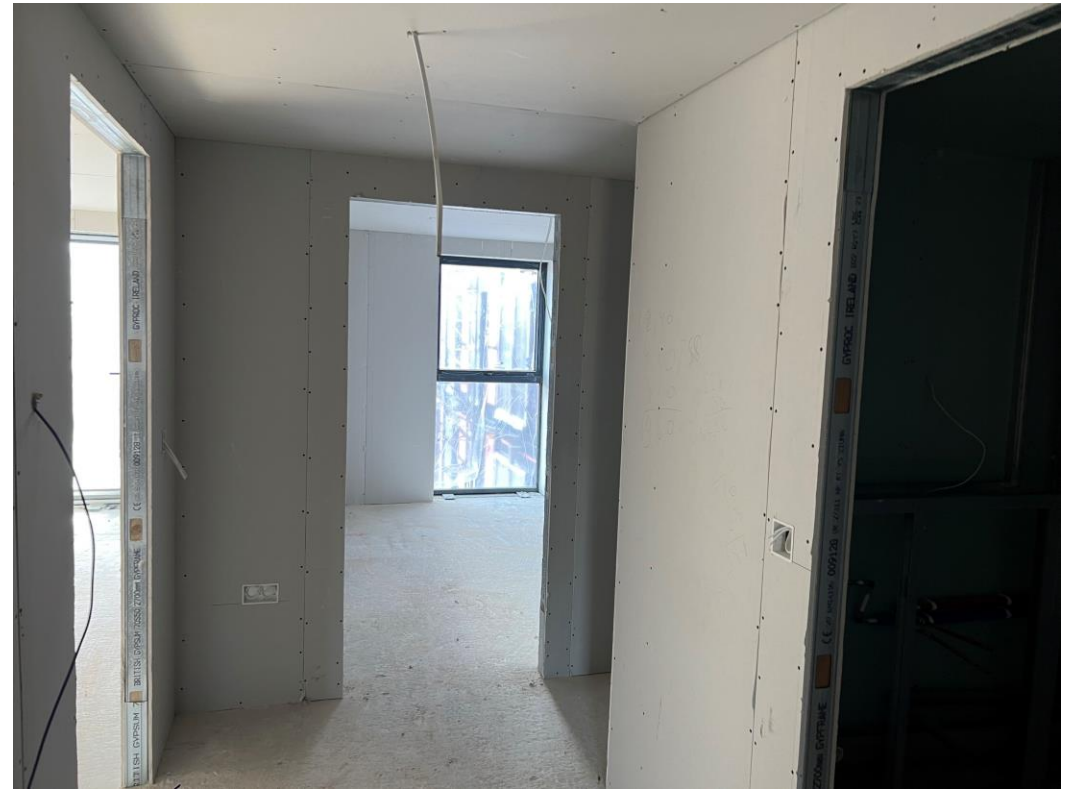
Apartment ready for plaster skim
