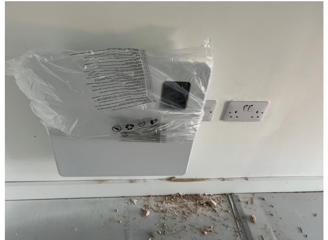
2 nd fix electrical
