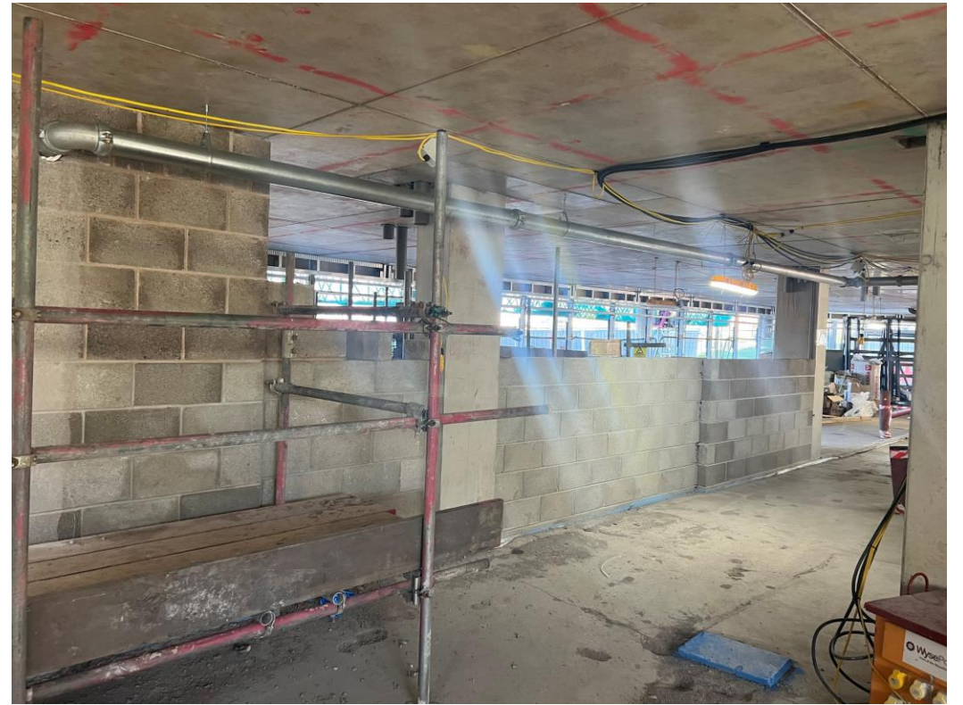
Ground level walls formed
