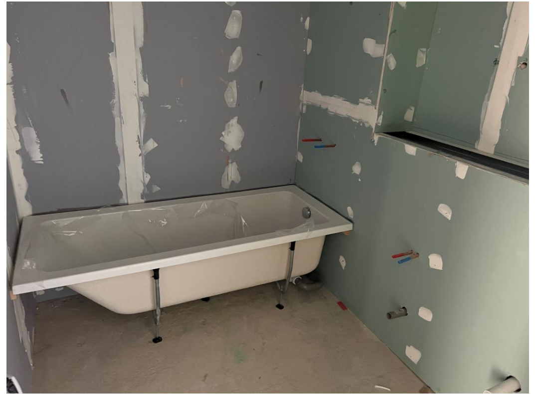
Sanitary installation commenced
