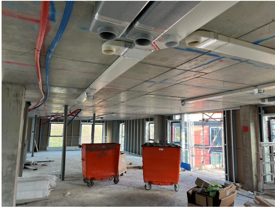
Upper level 1 st fix mechanical ducting & water
