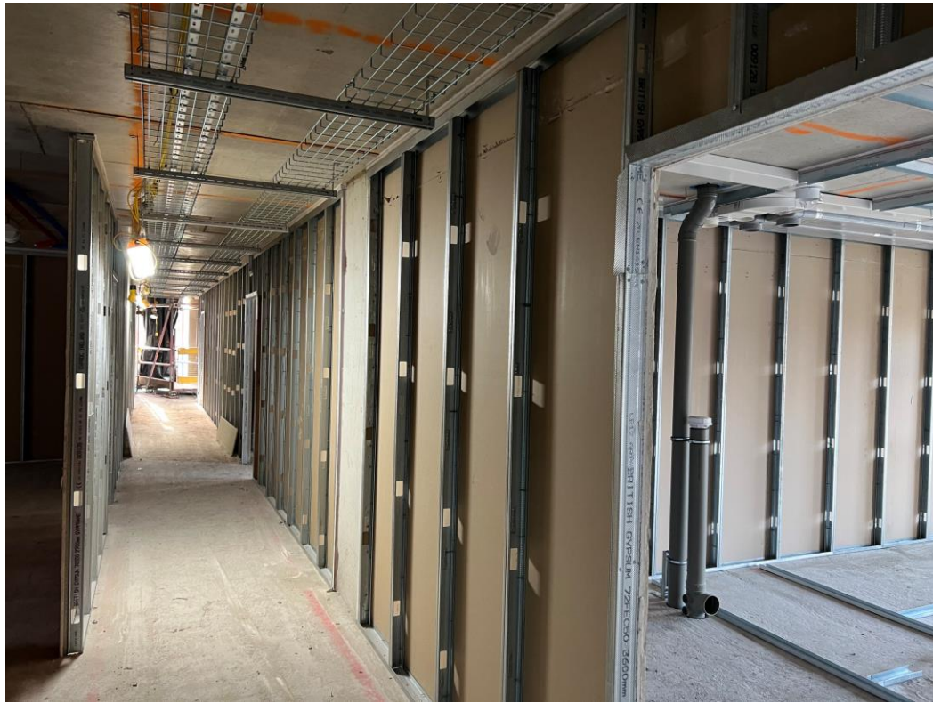
1 st Floor partition walls
