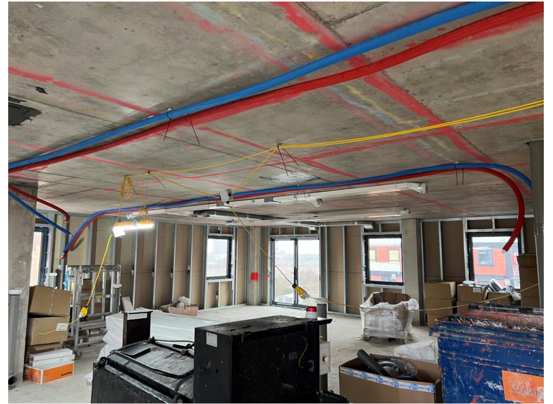
6 th Floor external walls and windows installed
