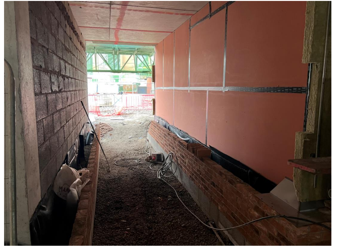
Block B facing brickwork
