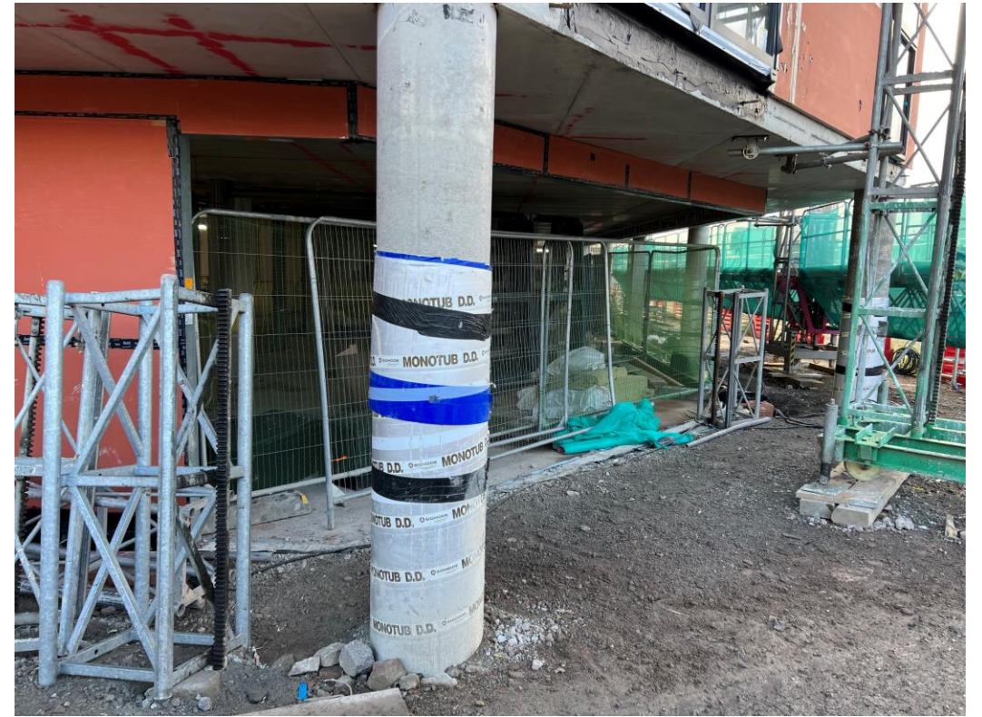
Block A Entrance
