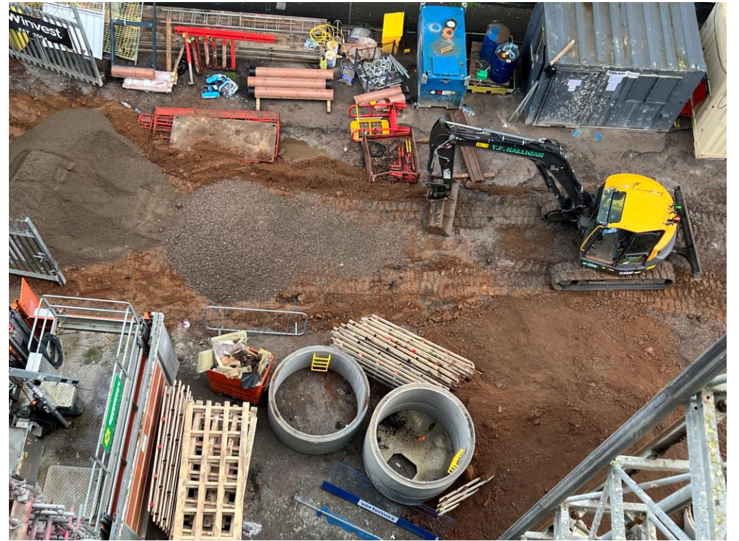
Underground drainage Dyer Street
