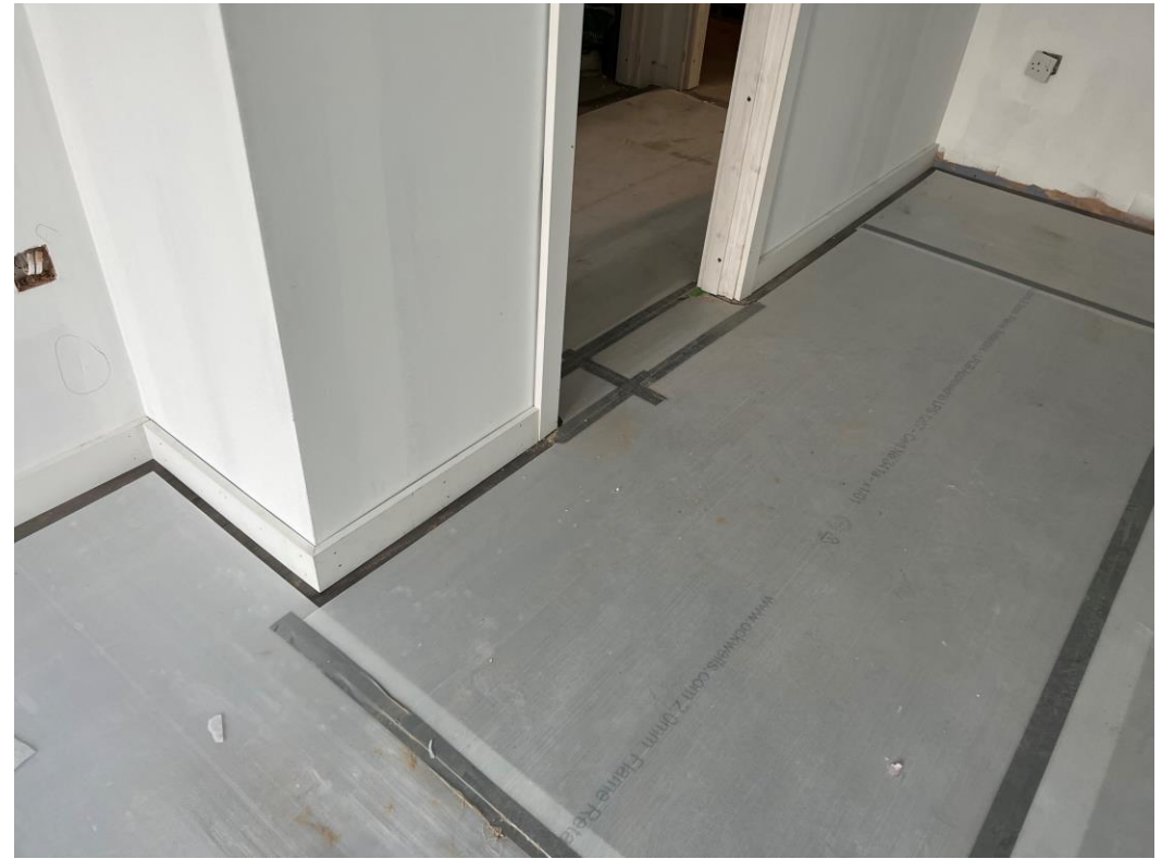
Apartment skirting and architraves
