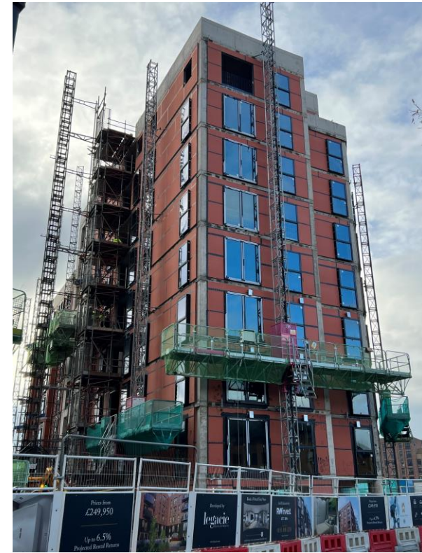
Ordsall Lane site view
