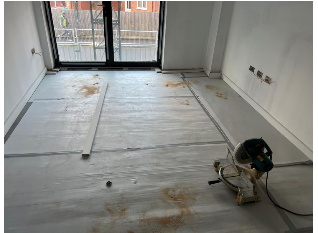
Apartment skirting and architraves
