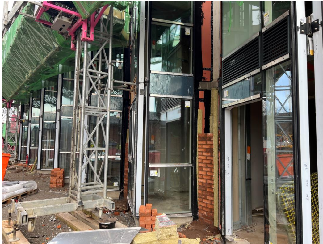
Block B facing brickwork
