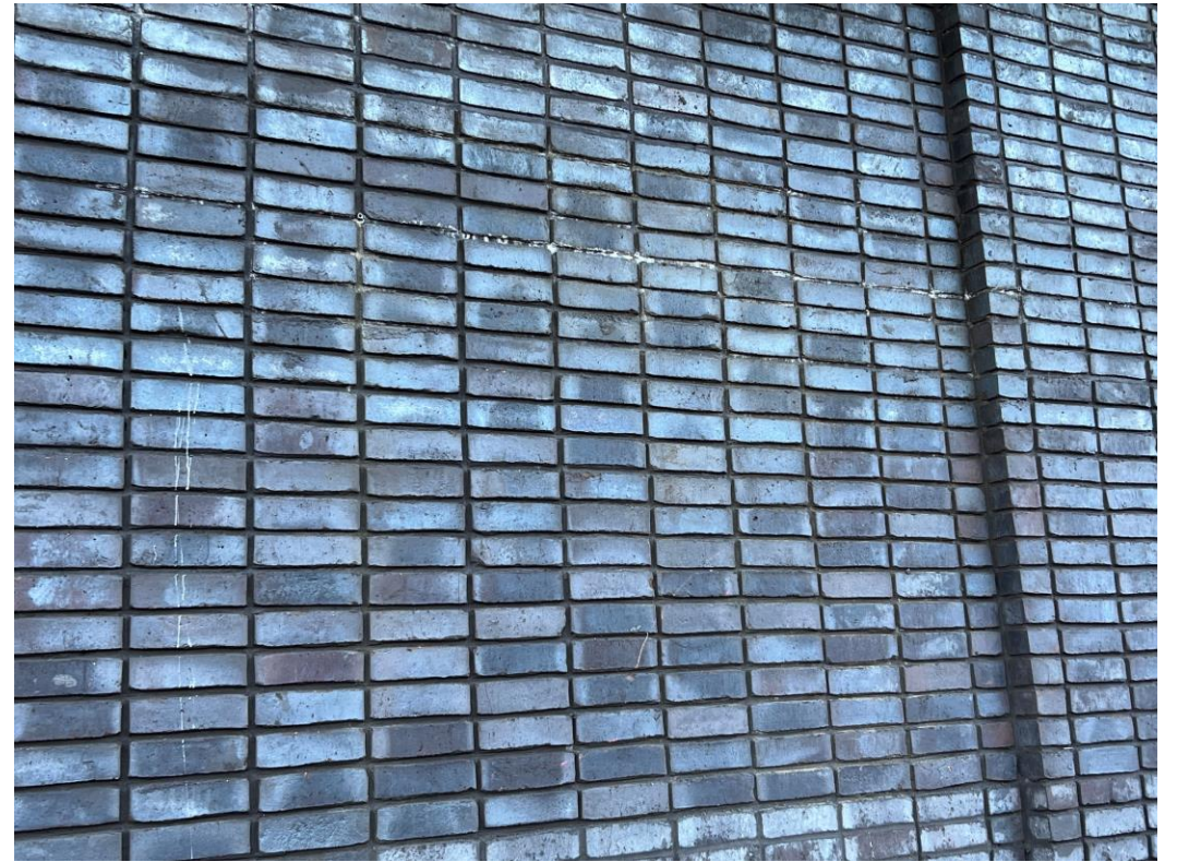
Block B facing brickwork
