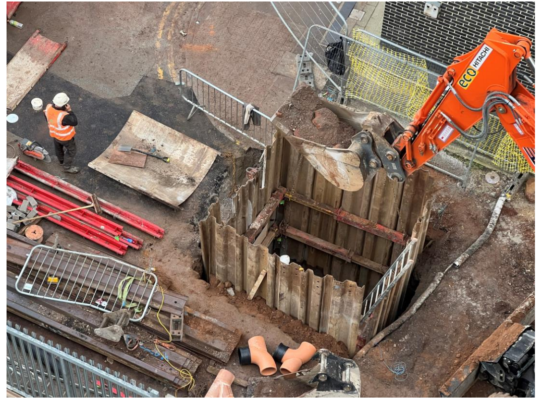
Underground drainage Dyer Street
