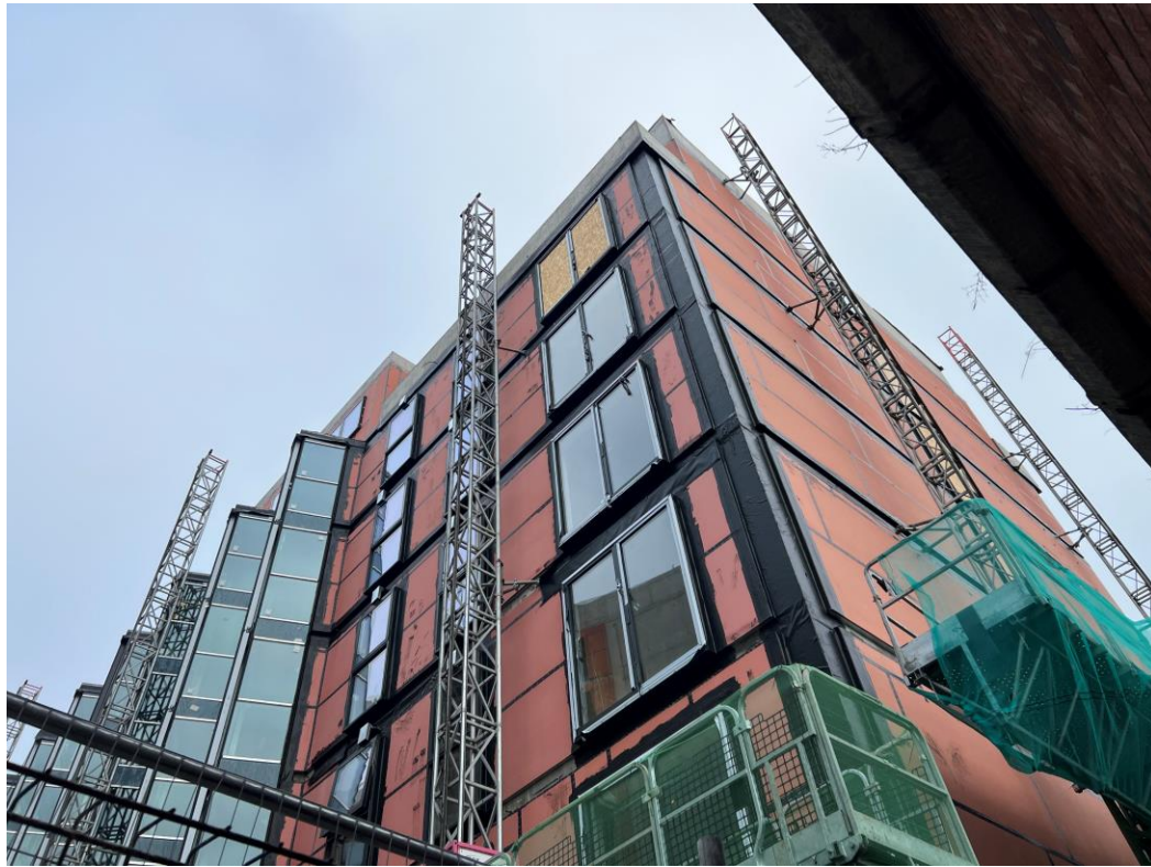
Block B weatherboarding & windows installed
