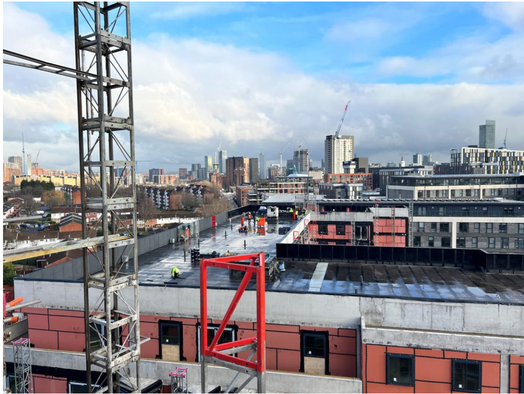
Block B roof covering
