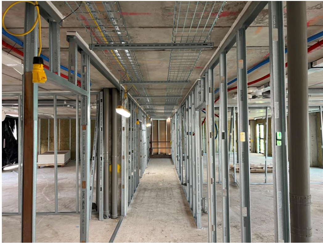
2 nd Floor partition walls
