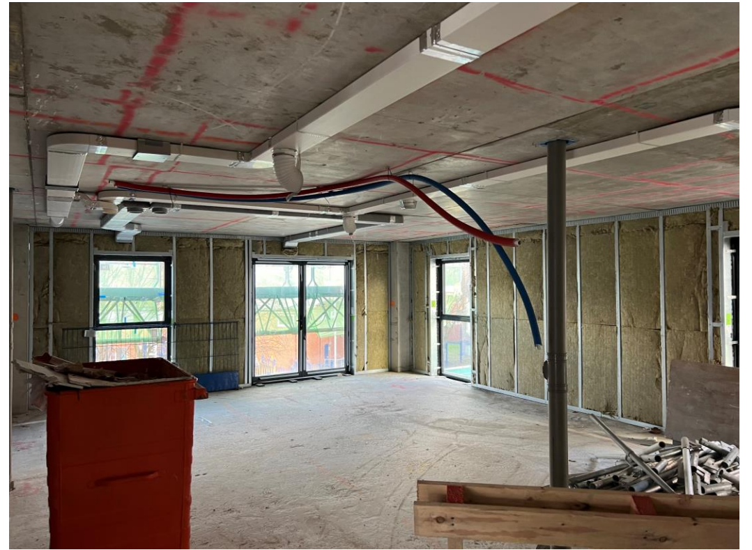
2 nd Floor partition walls
