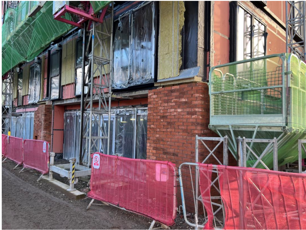
Block B facing brickwork
