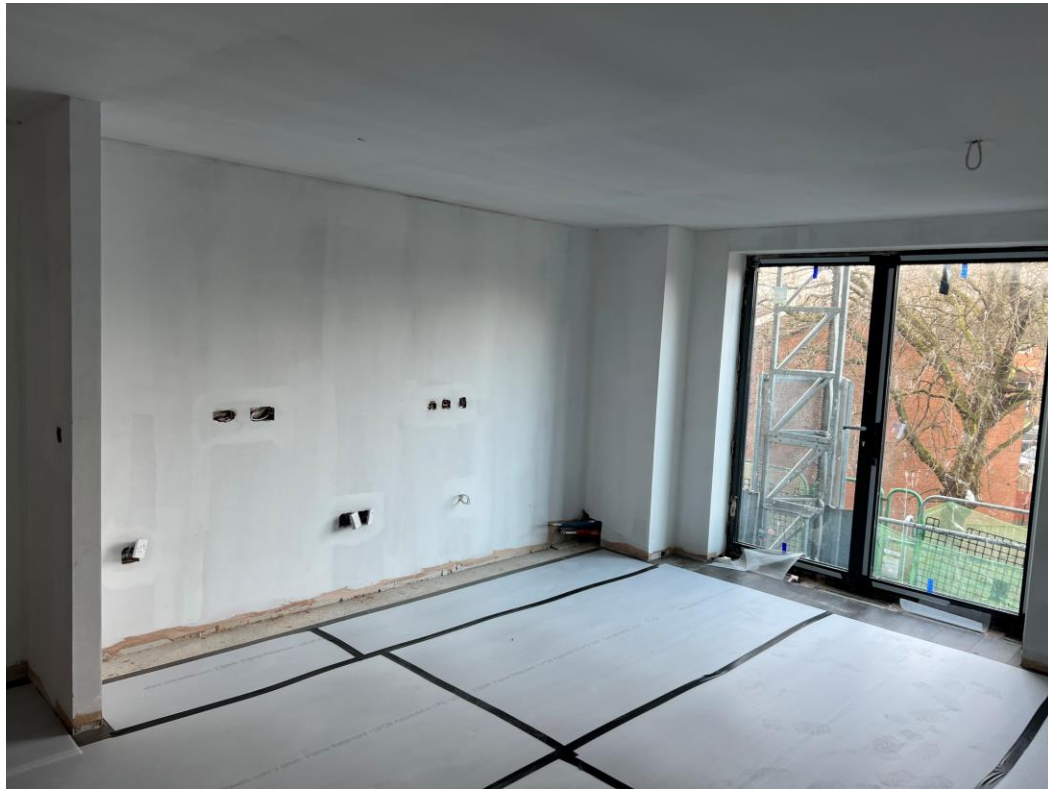
Apartment decoration commenced
