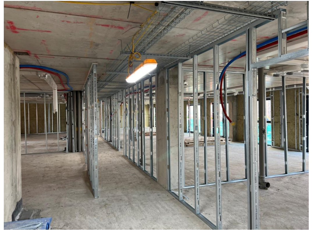
2 nd Floor partition walls
