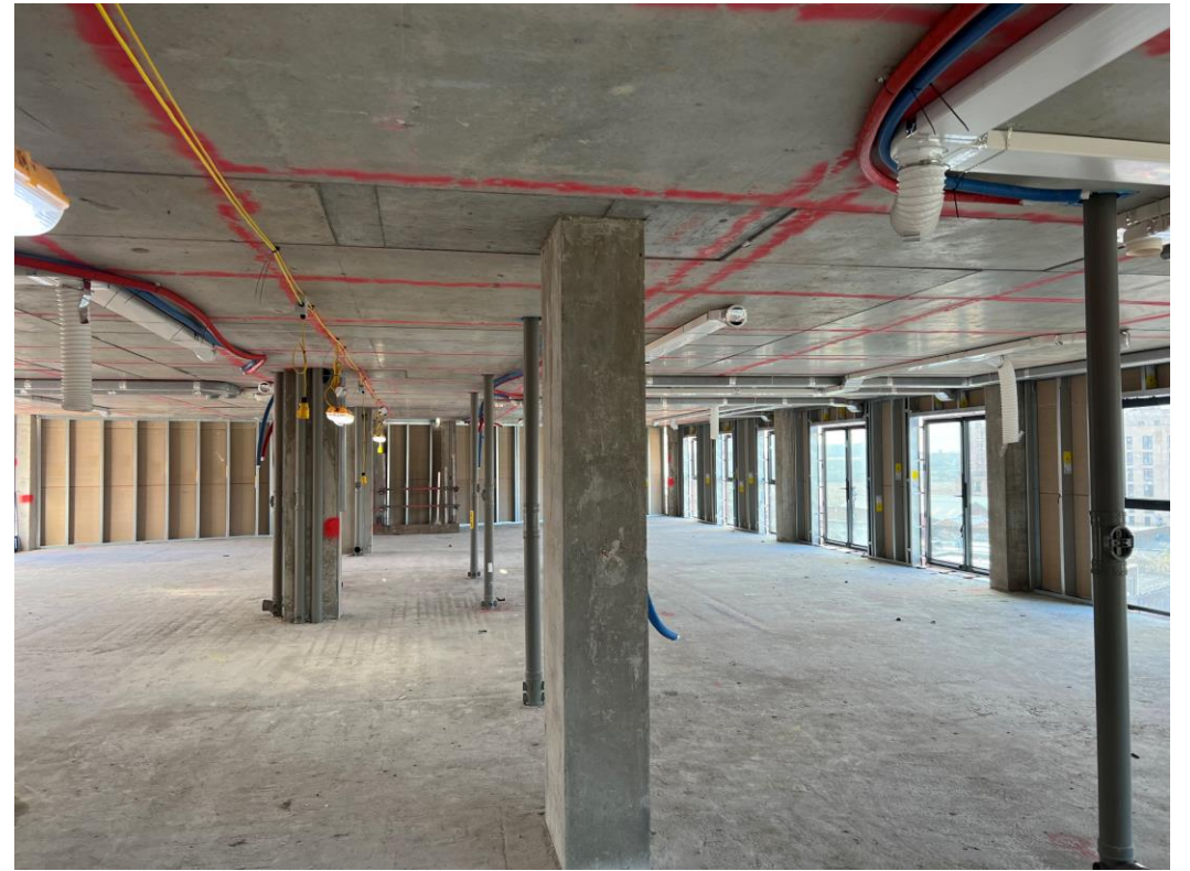
Upper level 1 st fix mechanical ducting & water
