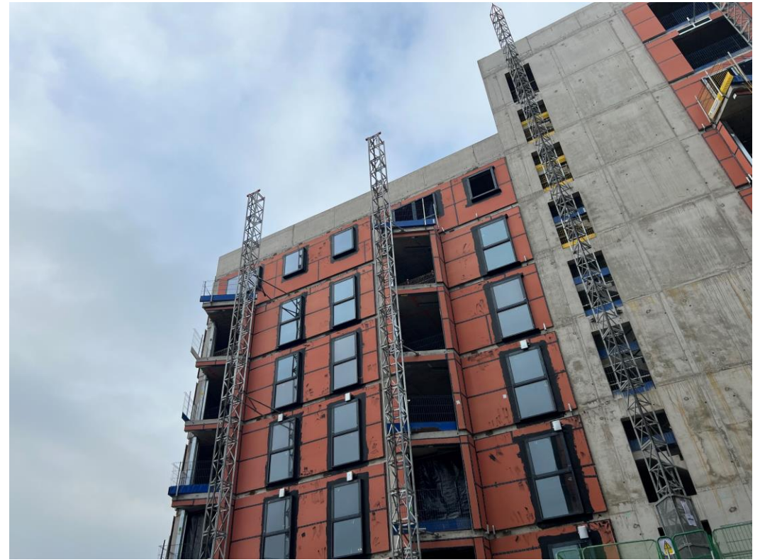
Block A weatherboarding & windows installed
