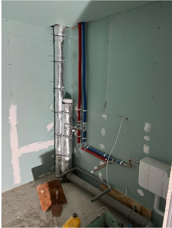
Apartment 1 st fix sanitary
