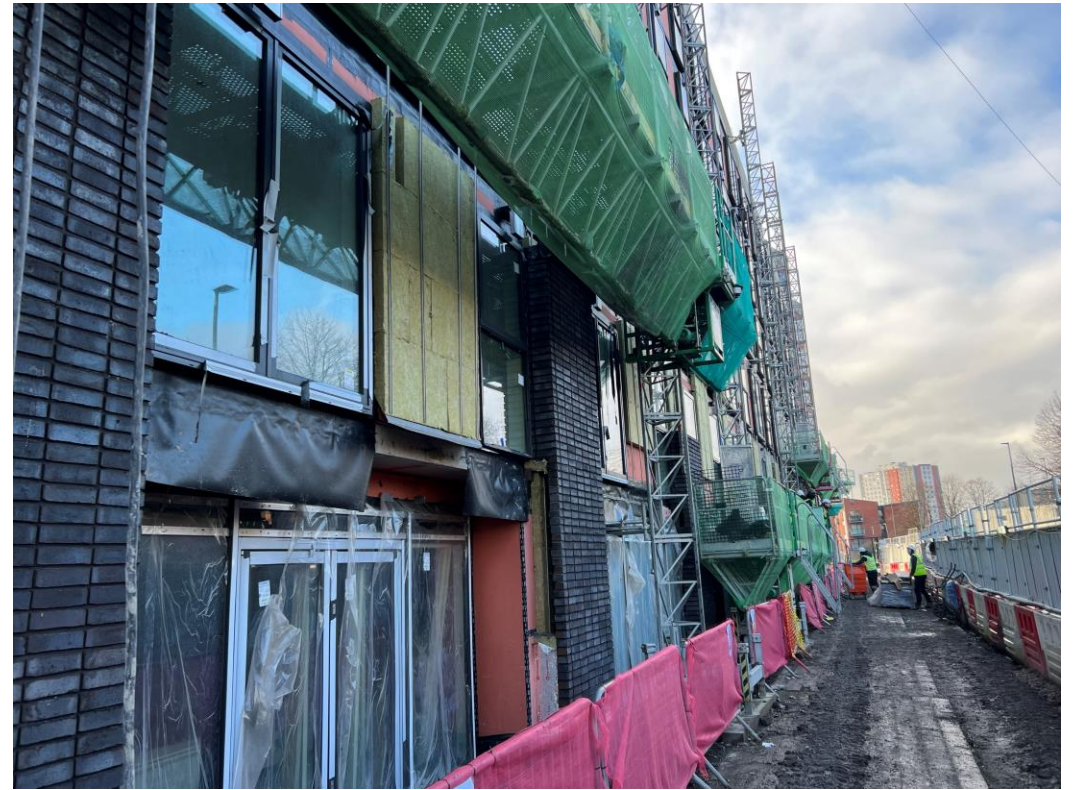
Block B facing brickwork
