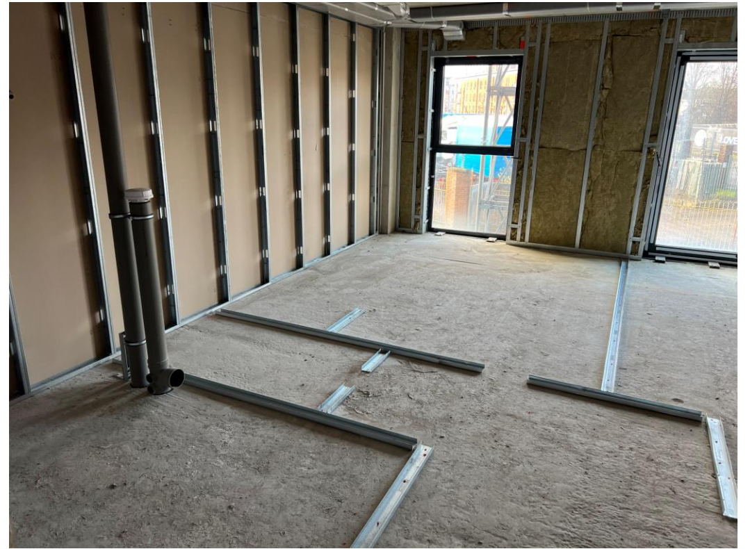
1 st Floor partition walls
