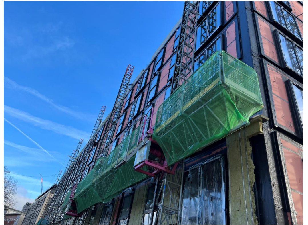
Block B wall insulation installed
