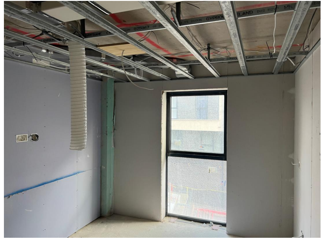
Upper floor Apartment partitions formed
