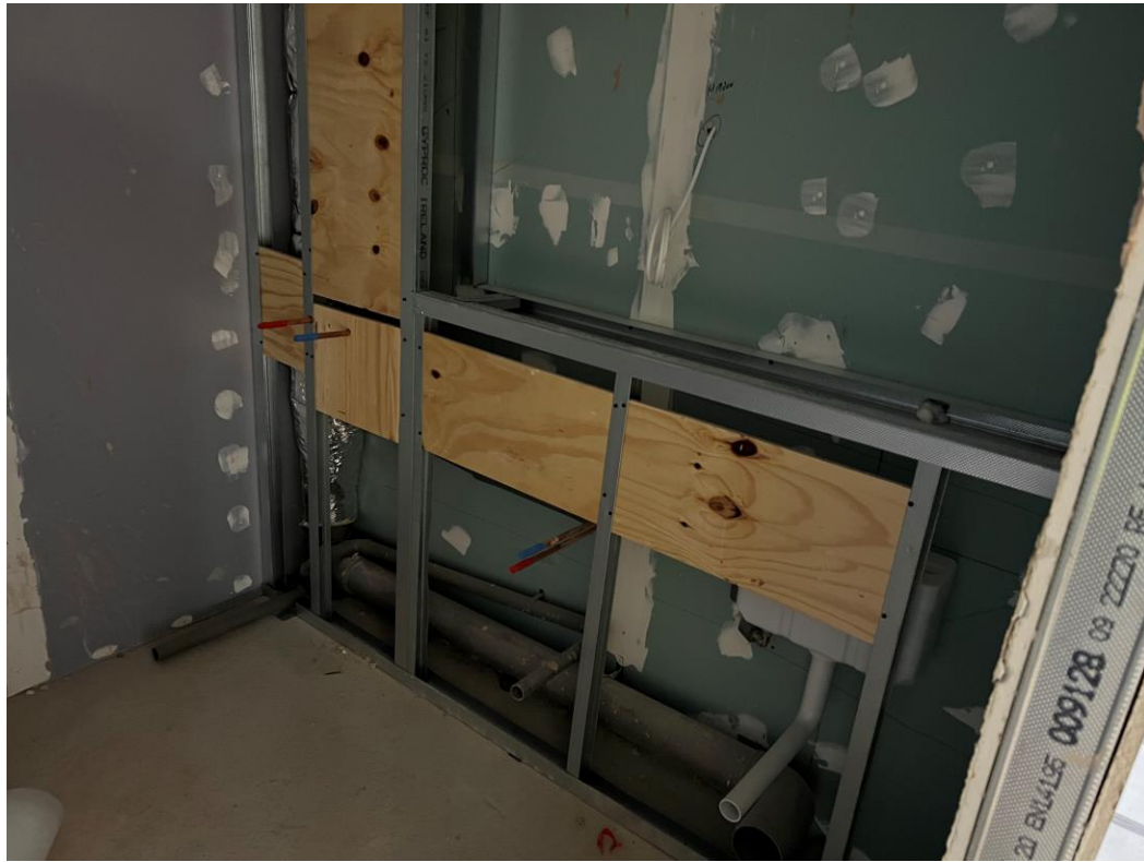
Apartment 1 st fix sanitary
