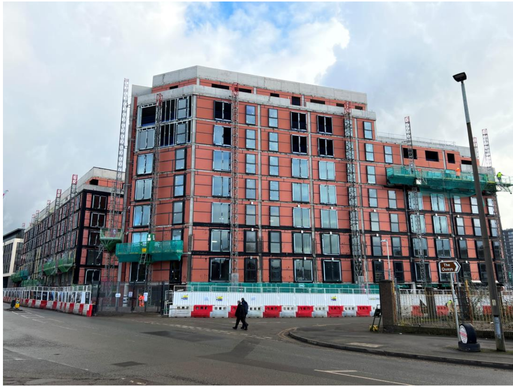
Ordsall Lane site view
