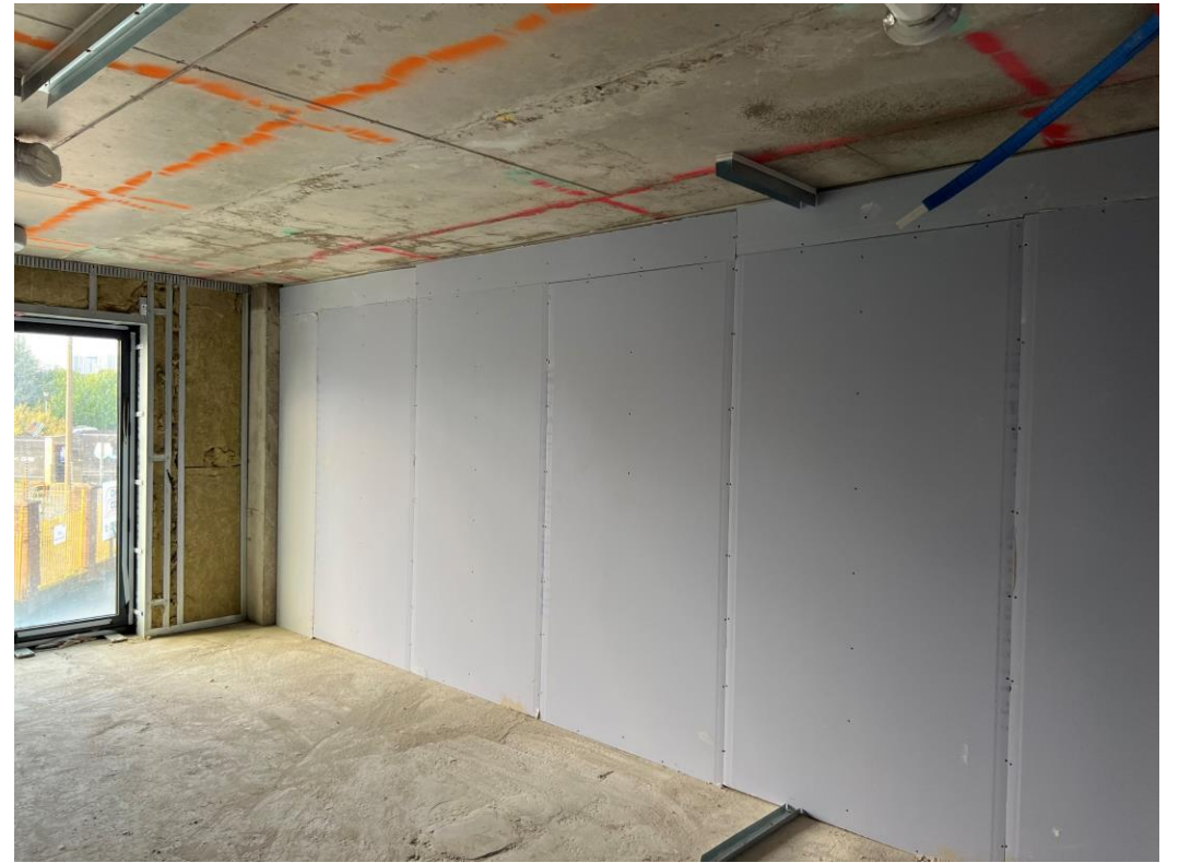
1 st Floor partition walls
