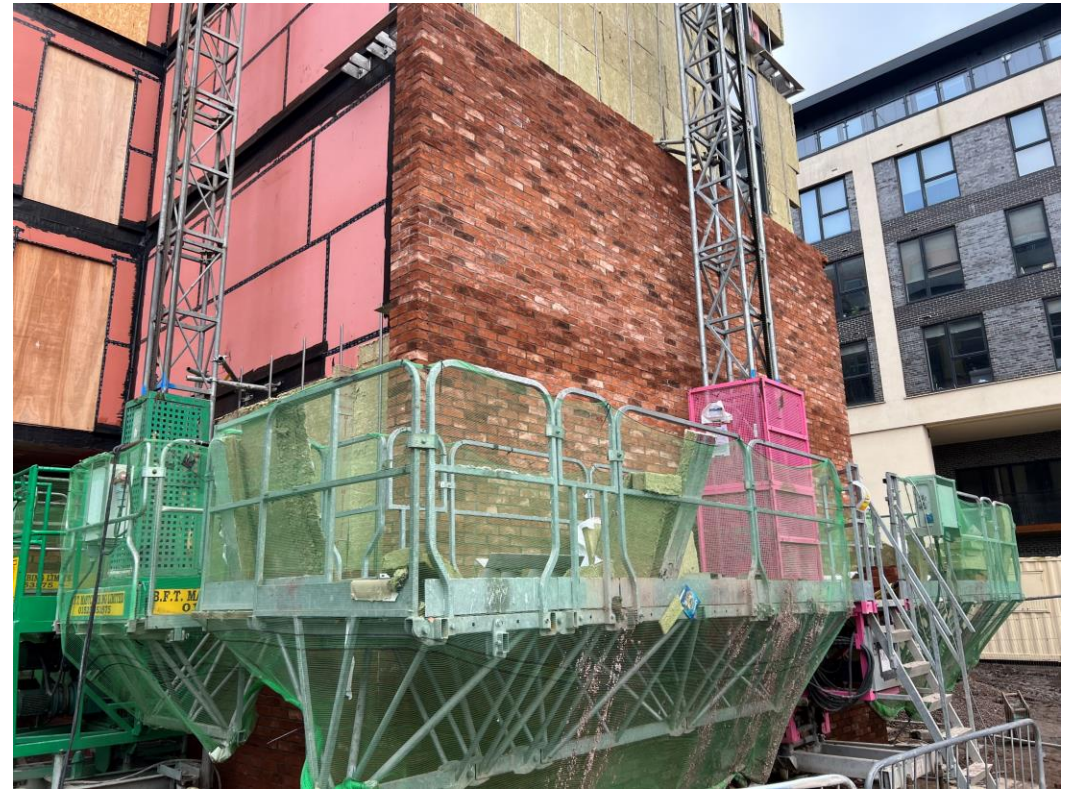
Block B facing brickwork
