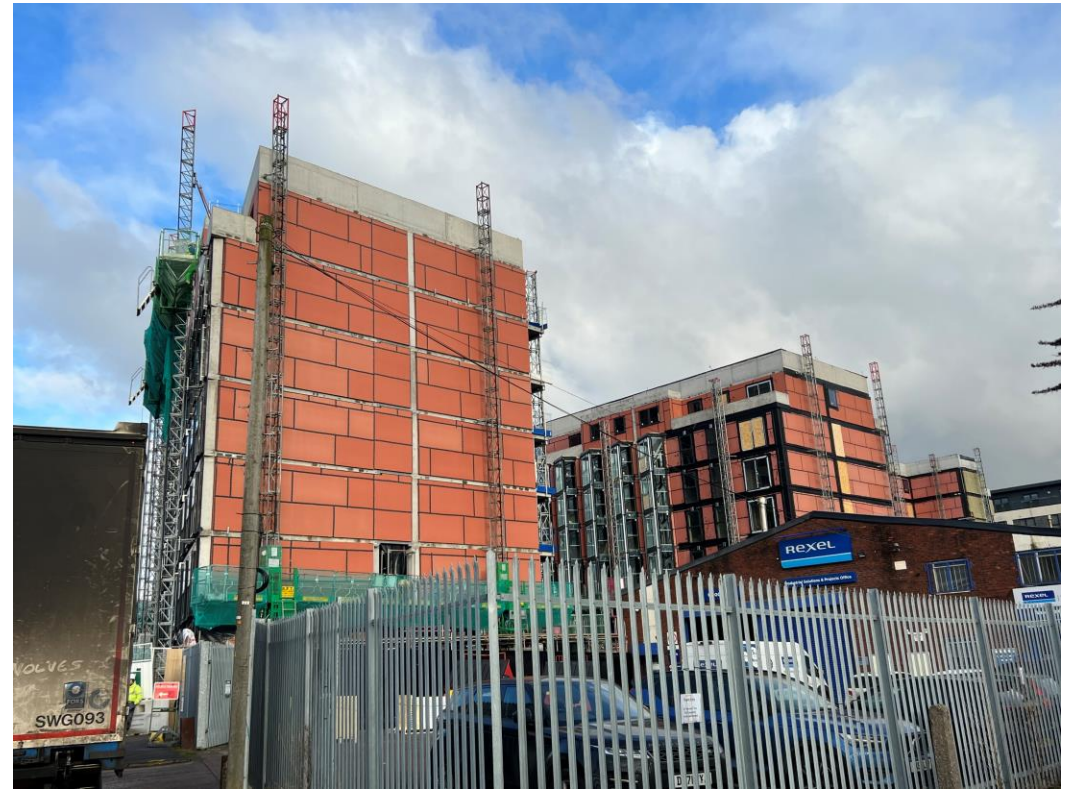
Worrall Street site view
