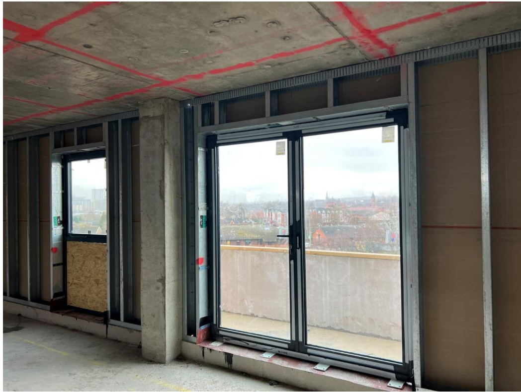
6 th Floor external walls and windows installed
