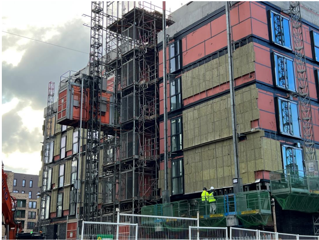
Ordsall Lane site view
