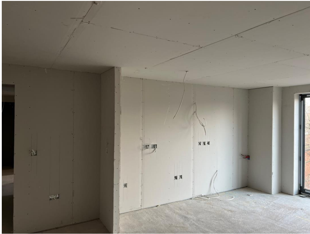
Apartment prepared for plaster skim
