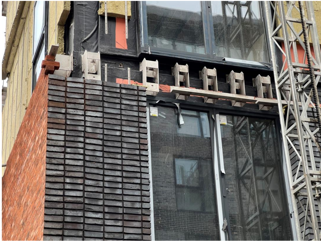
Block B facing brickwork
