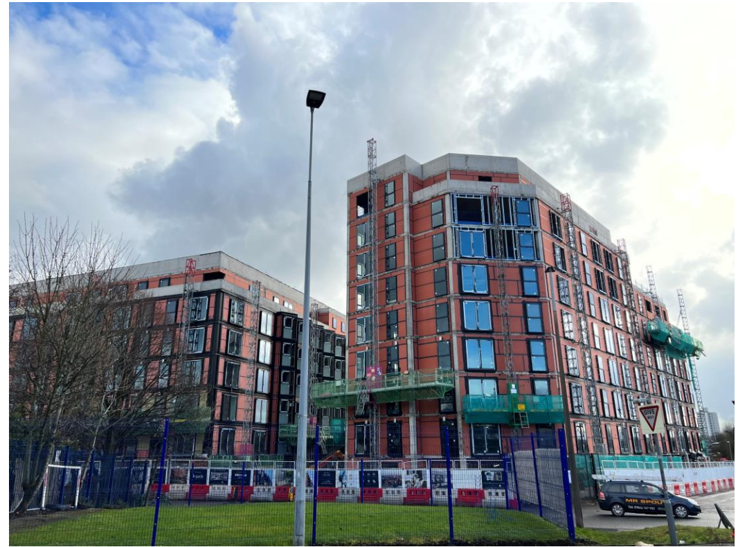
Ordsall Lane site view
