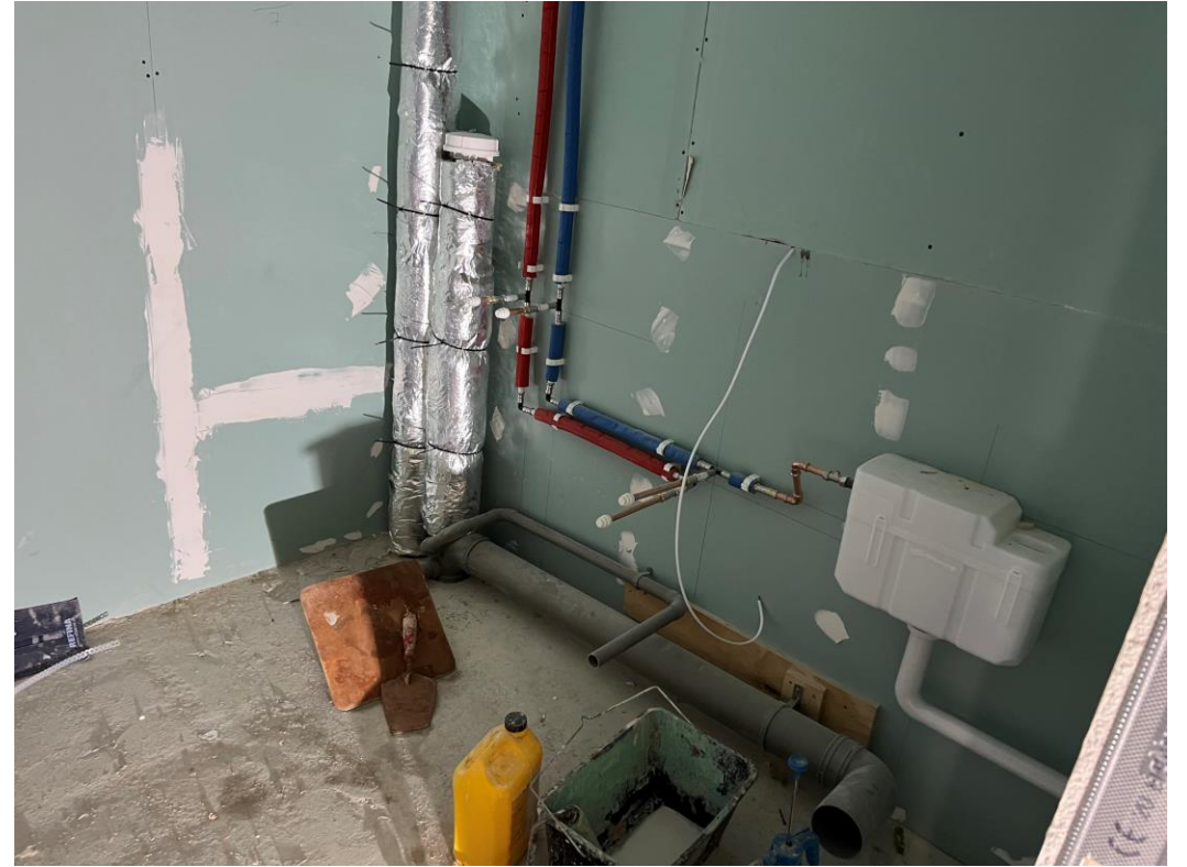
Apartment 1 st fix sanitary
