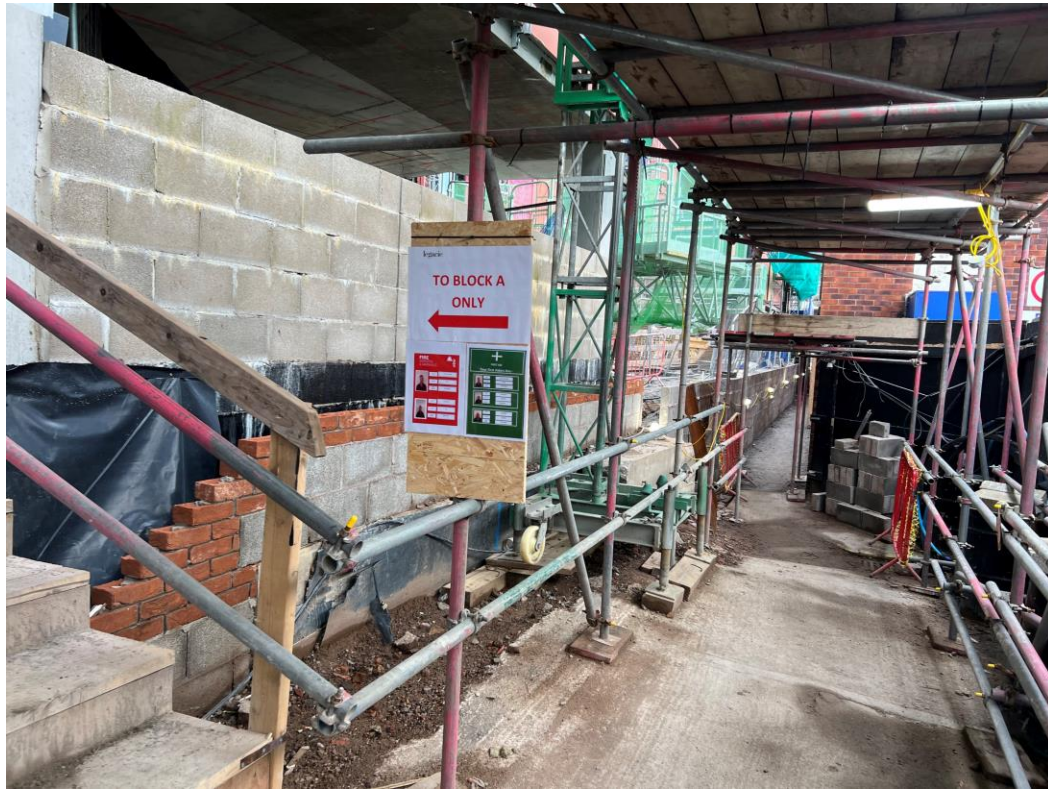
Block A facing brickwork
