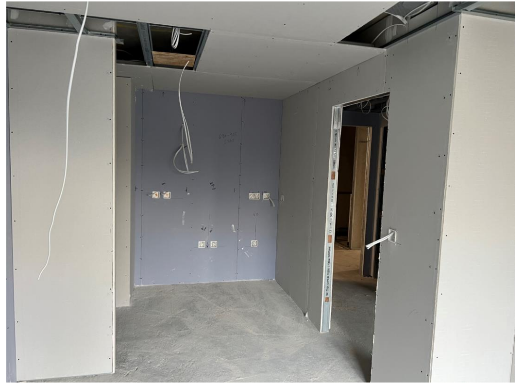
Apartment prepared for plaster skim
