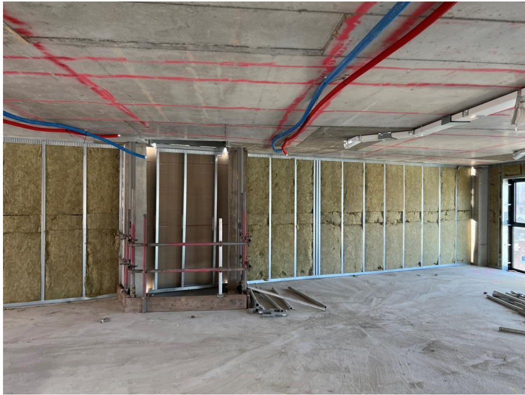
Upper level 1 st fix mechanical ducting & water
