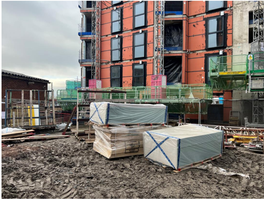
Block A weatherboarding & windows installed
