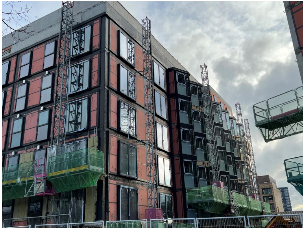
Ordsall Lane site view
