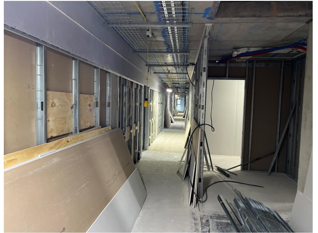
Upper floor Apartment partitions formed
