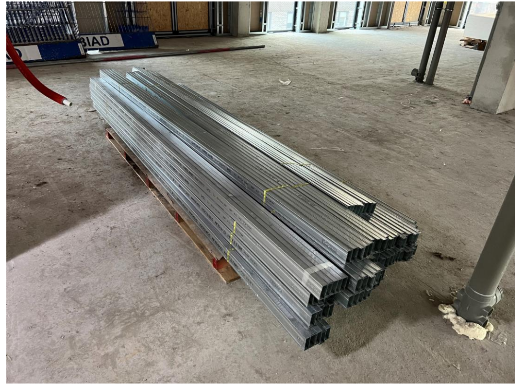
5 th Floor partition wall materials
