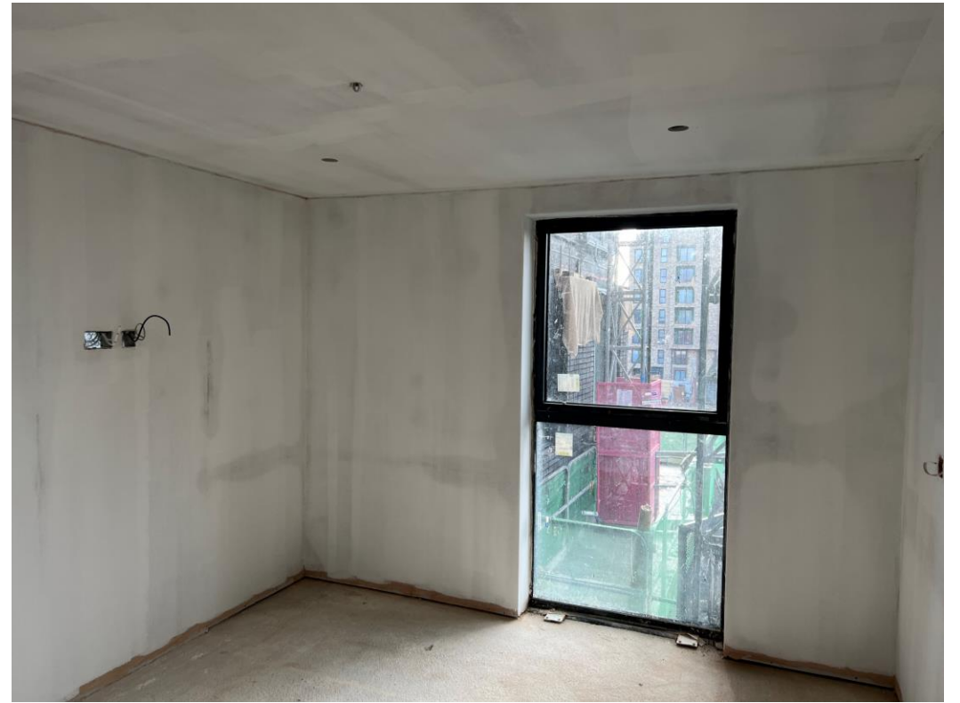
Apartment decoration commenced
