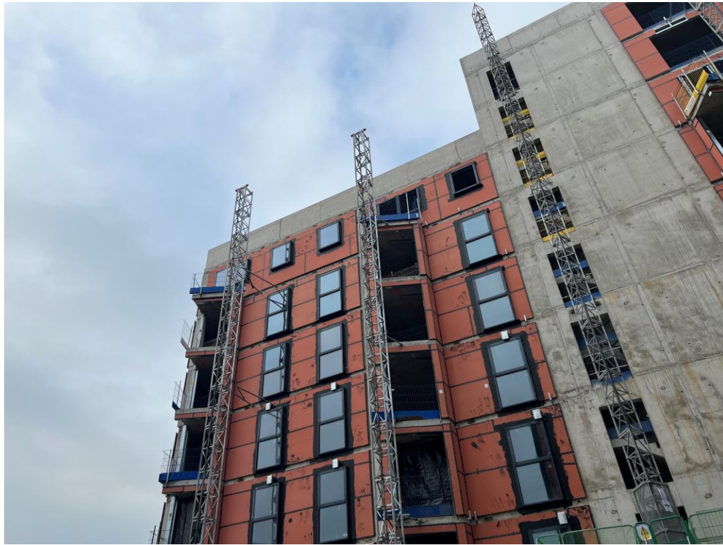
Block A weatherboarding & windows installed
