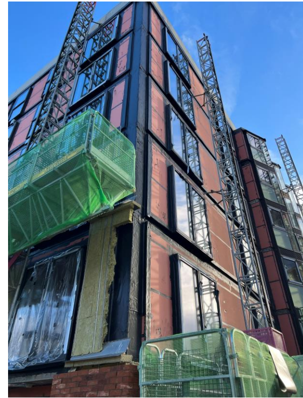
Block B weatherboarding & windows installed
