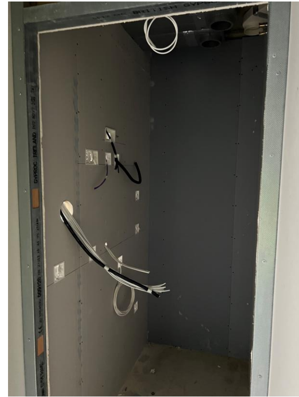
Apartment 1 st fix electrical
