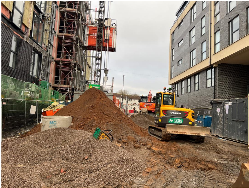
Underground drainage Dyer Street
