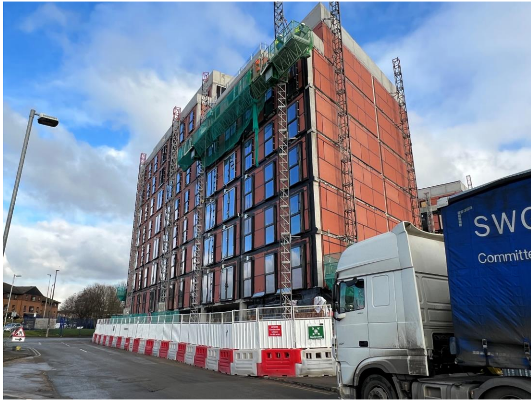
Worrall Street site view
