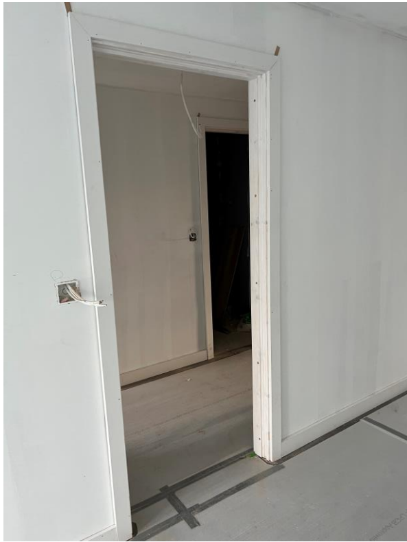
Apartment skirting and architraves
