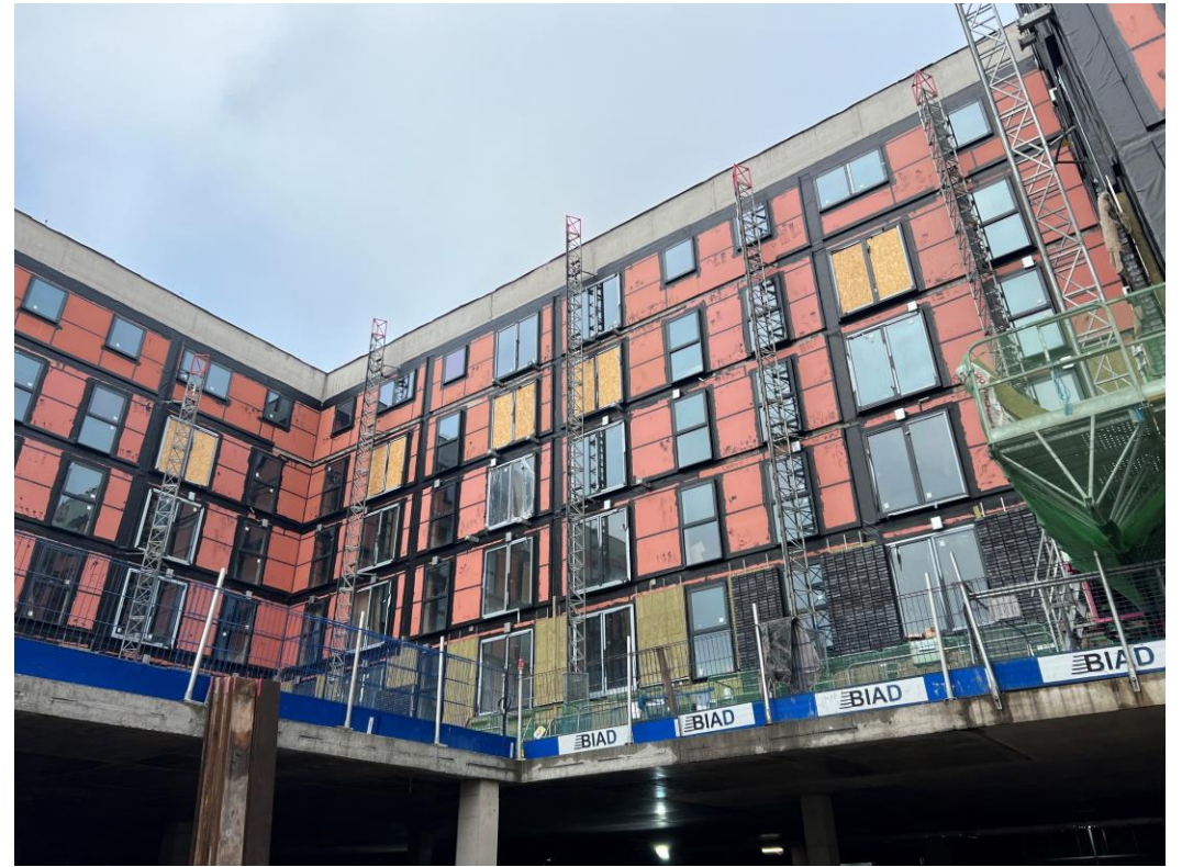
Block B facing brickwork
