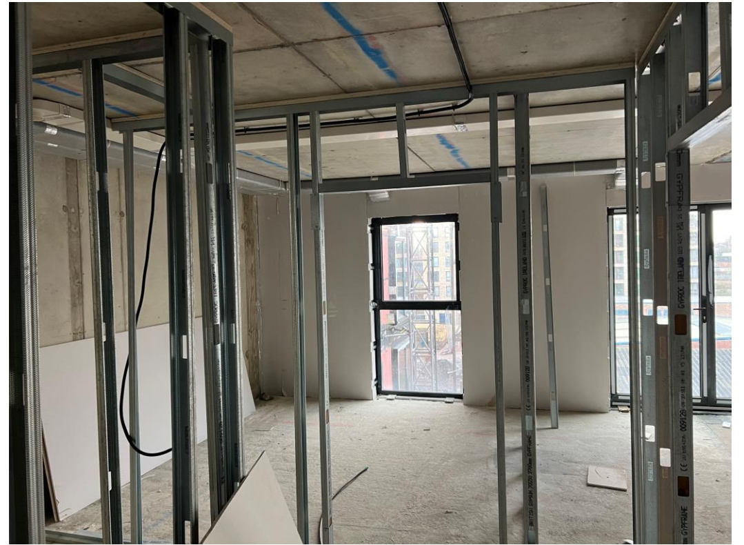
Upper floor Apartment partitions formed
