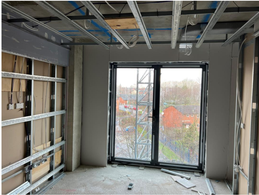
Upper floor Apartment partitions formed
