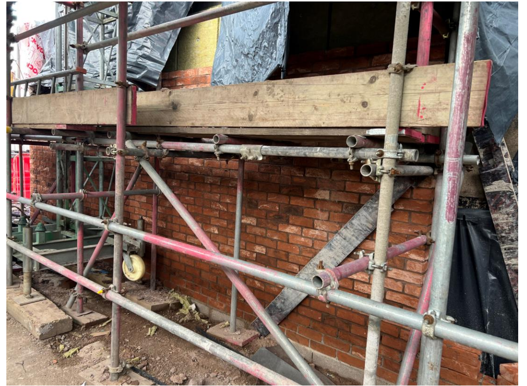
Block A facing brickwork
