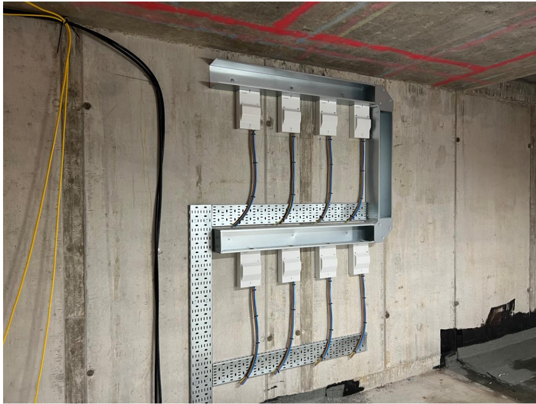
6 th Floor 1 st Fix electrical meter supply
