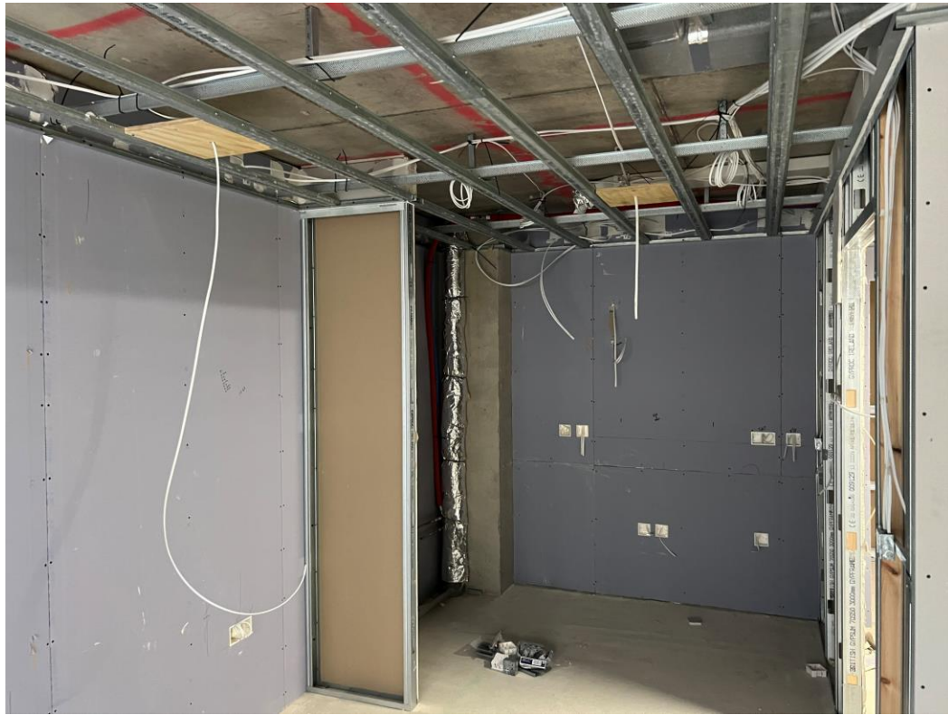
Upper floor Apartment partitions formed
