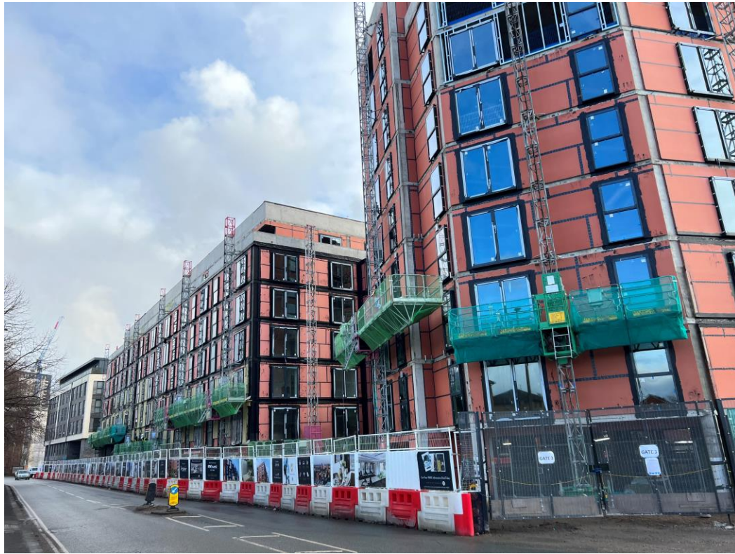
Ordsall Lane site view
