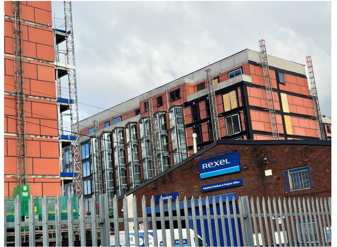
Worrall Street site view
