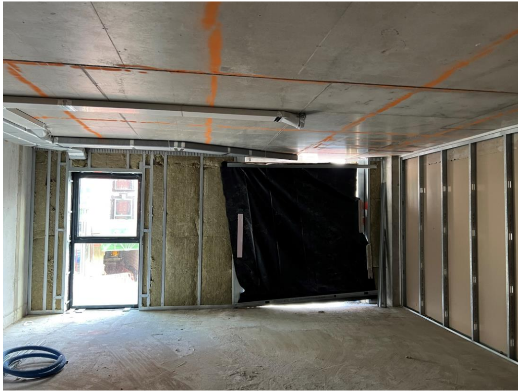
1 st Floor partition walls
