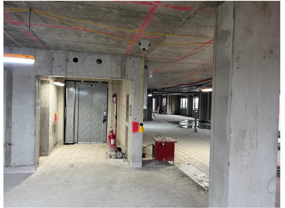
6 th Floor Lift installed
