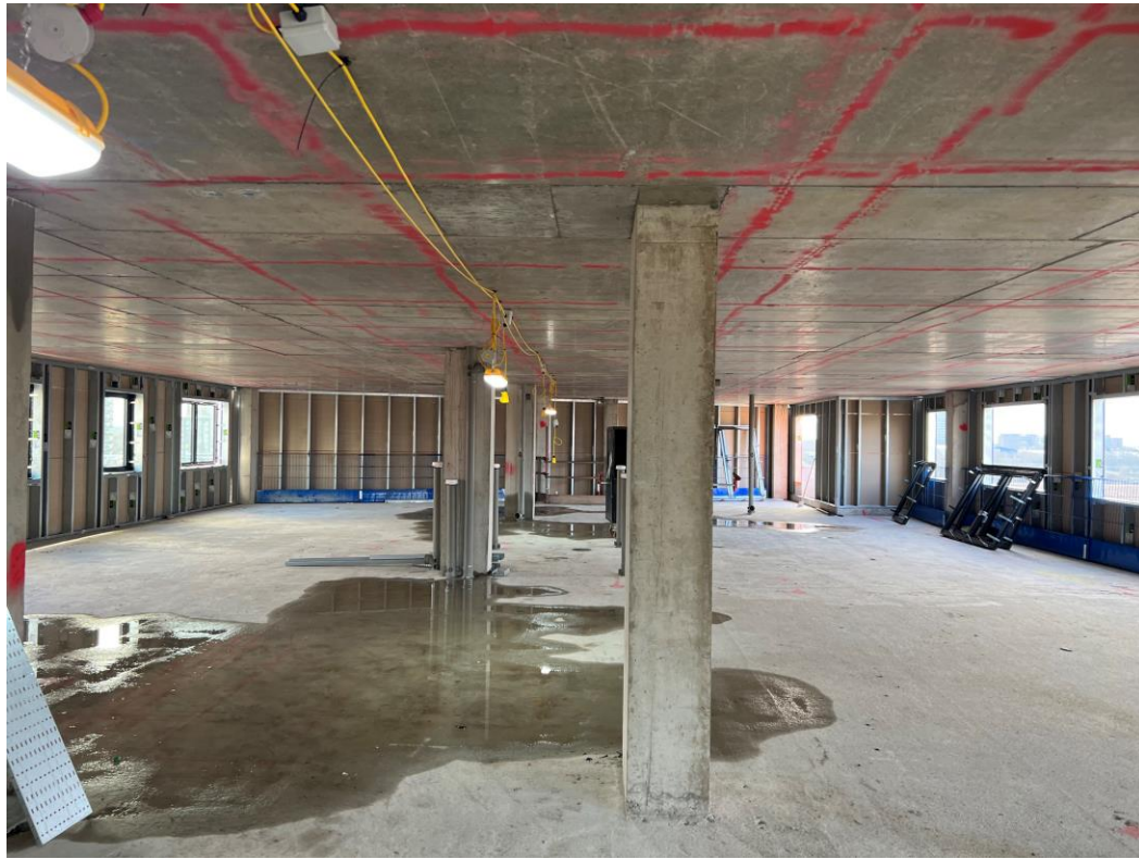
Upper level SFS & weatherboarding external walls
