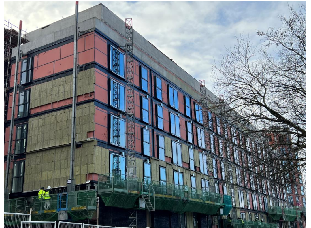
Ordsall Lane site view
