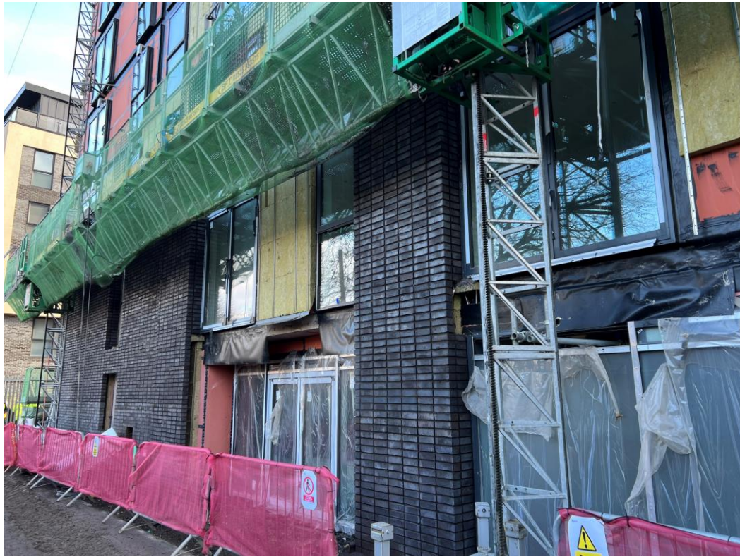
Block B facing brickwork
