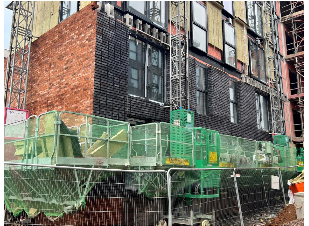
Block B facing brickwork
