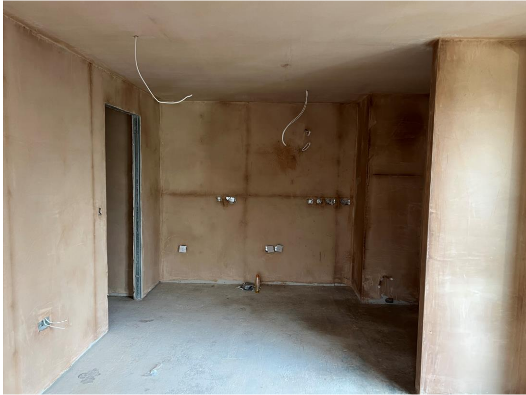
Upper level Apartment plaster skim ceiling and walls
