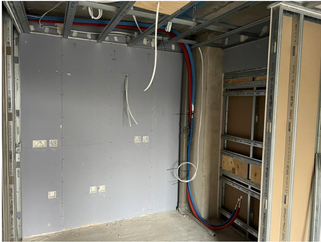
Apartment 1 st fix electrical
