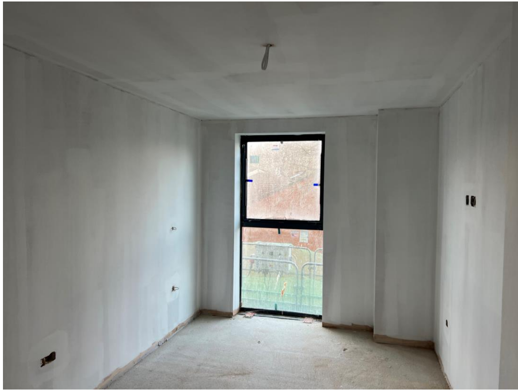
Apartment decoration commenced
