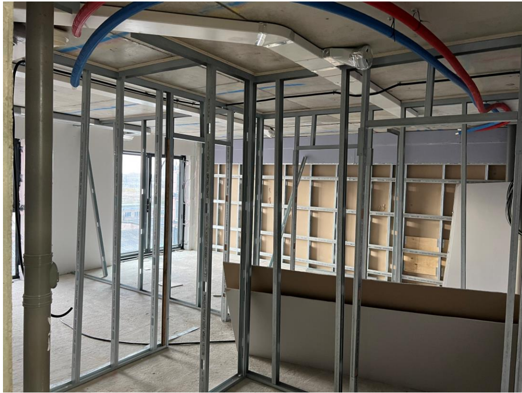
Upper floor Apartment partitions formed
