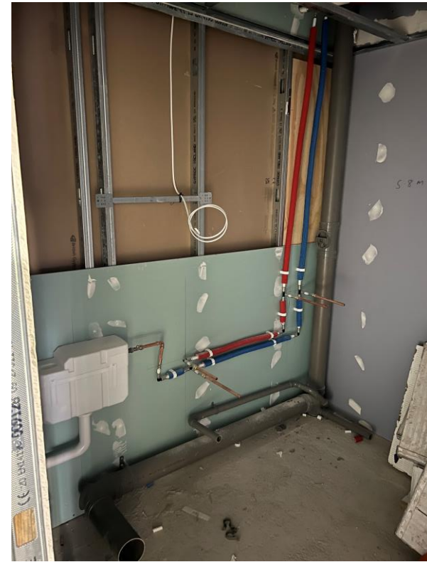
Apartment 1 st fix sanitary
