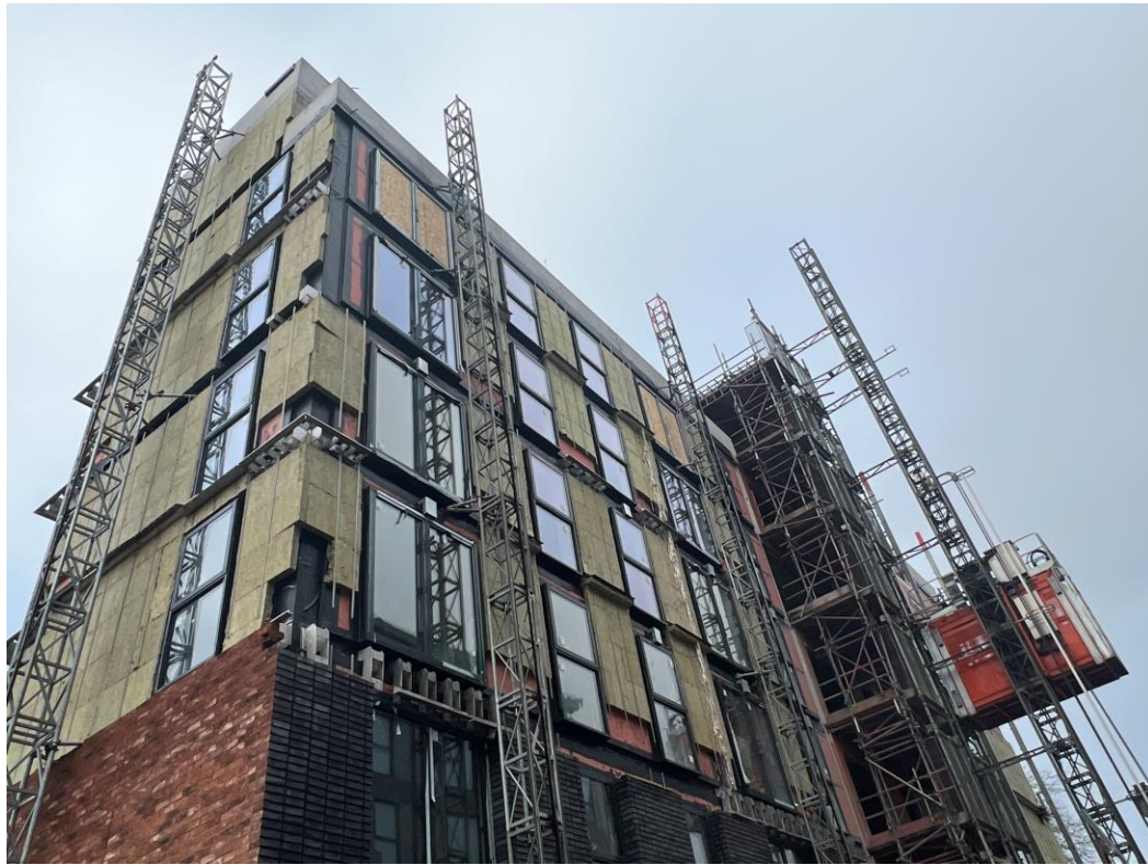
Block B facing brickwork
