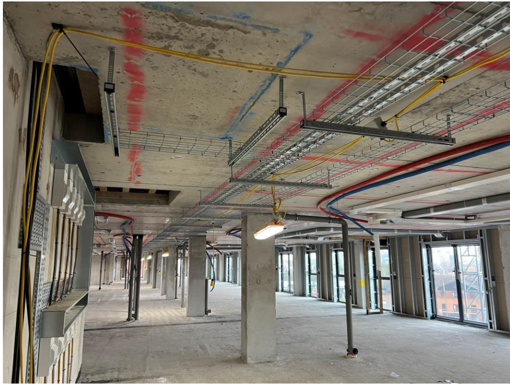
5 th Floor 1 st Fix electrical
