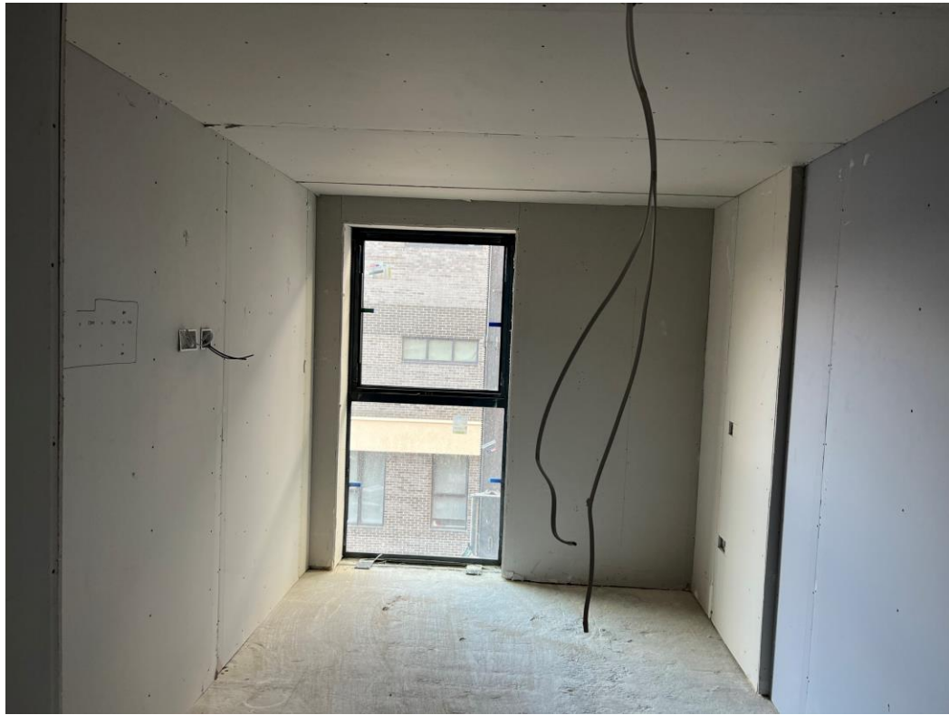
Apartment prepared for plaster skim
