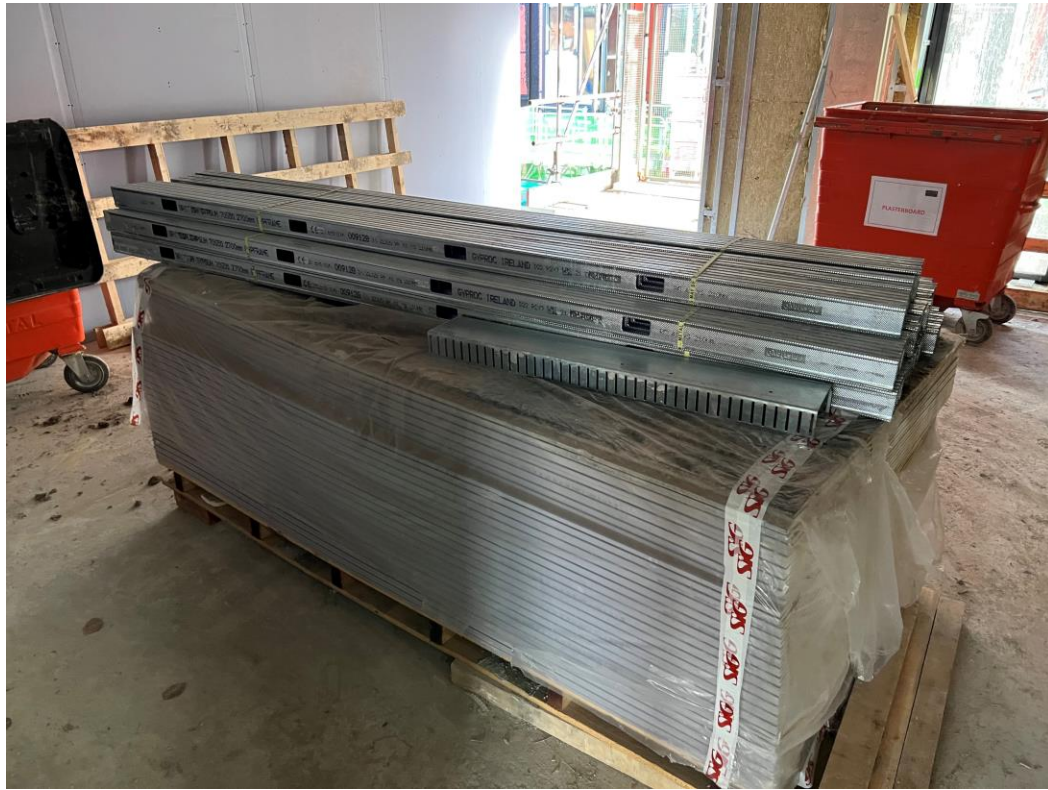
2 nd Floor partition walls
