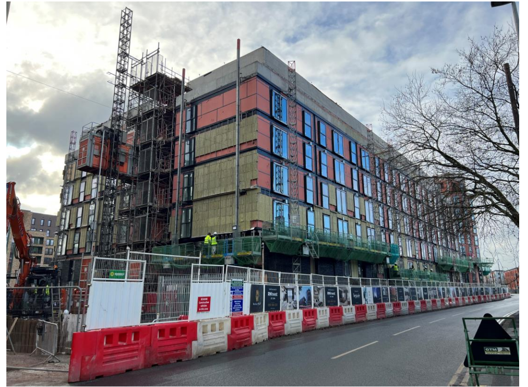
Ordsall Lane site view
