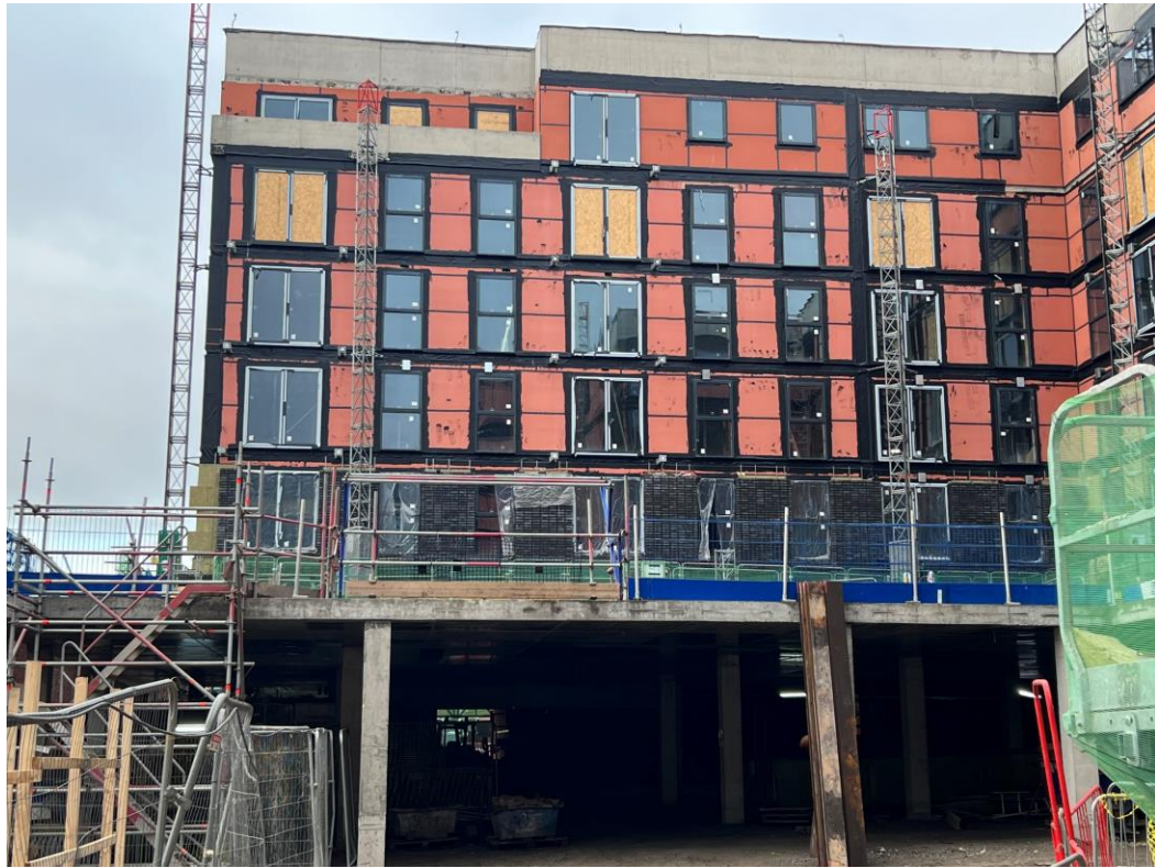
Block B facing brickwork
