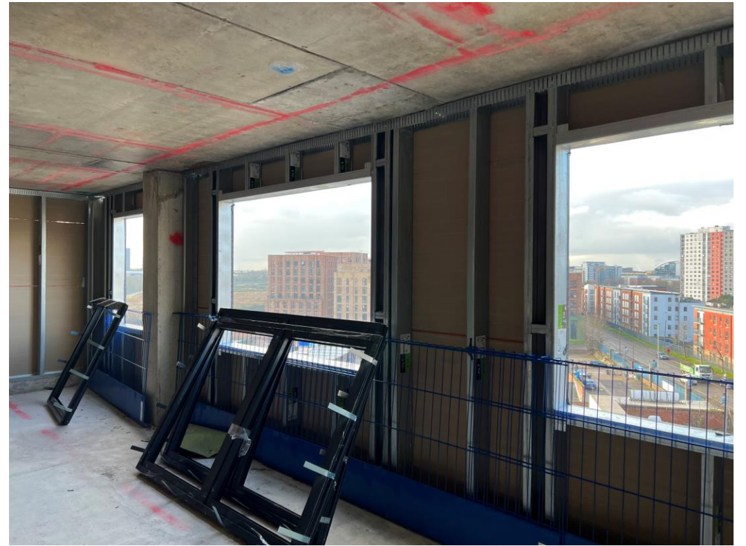
Upper level window installation
