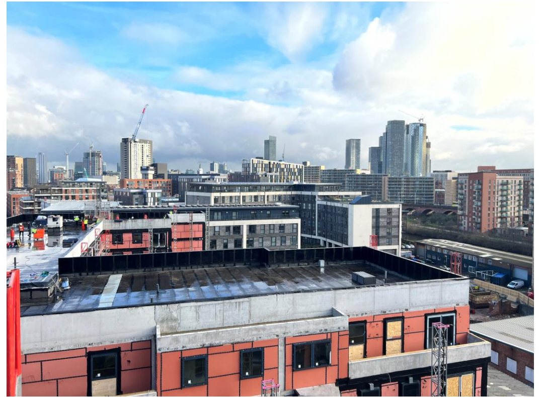
Block B roof covering
