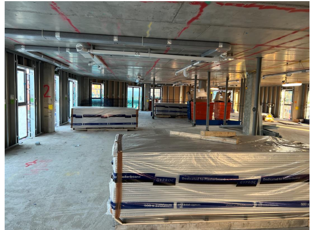
Upper level 1 st fix mechanical ducting
