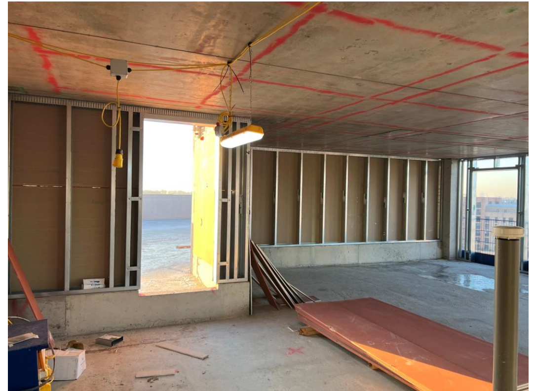
Upper level SFS and weatherboarding
