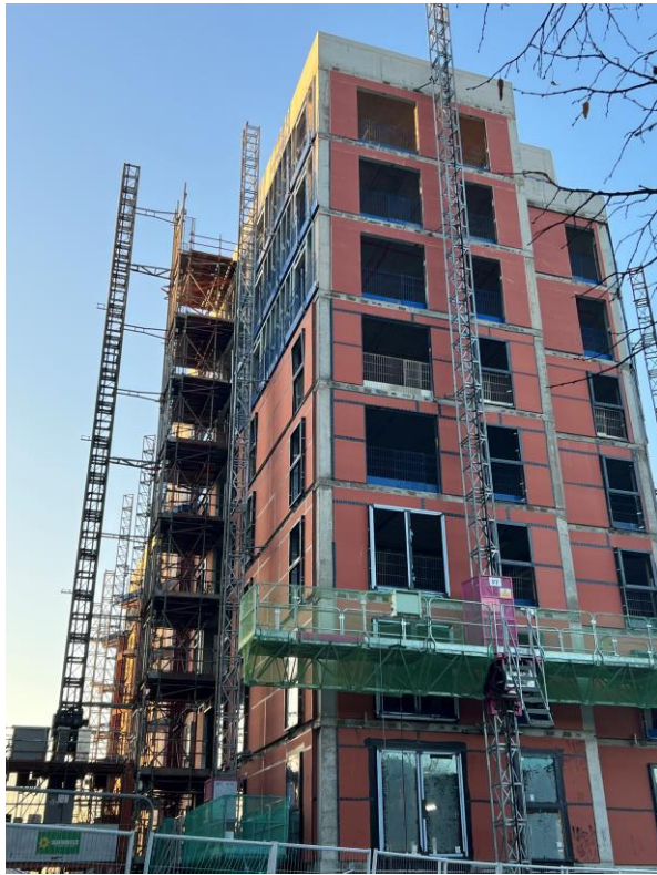
Ordsall Lane site view
