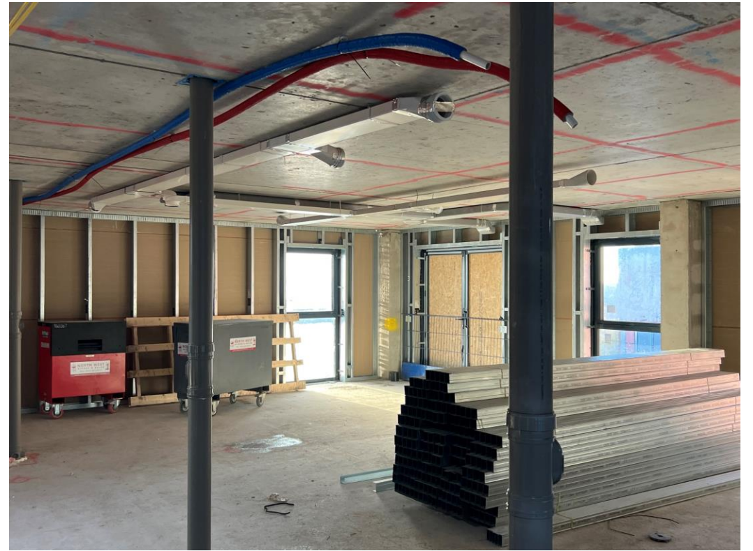
Upper levels hot and cold water supply
