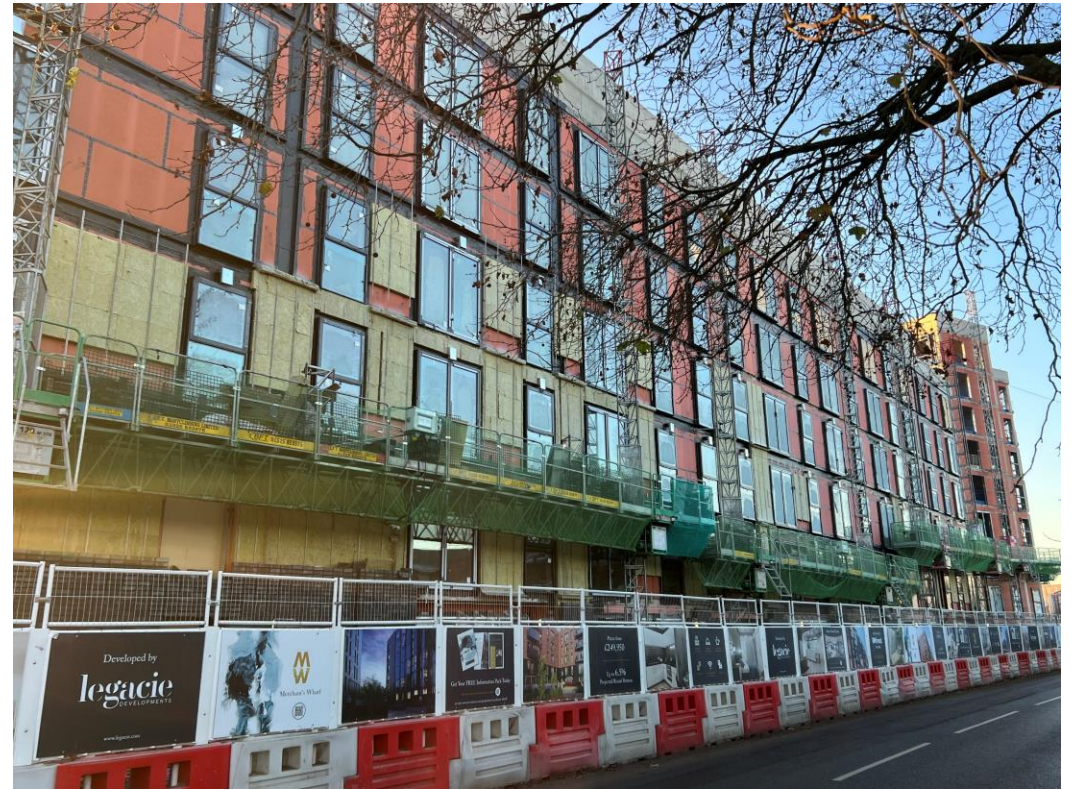
Ordsall Lane site view
