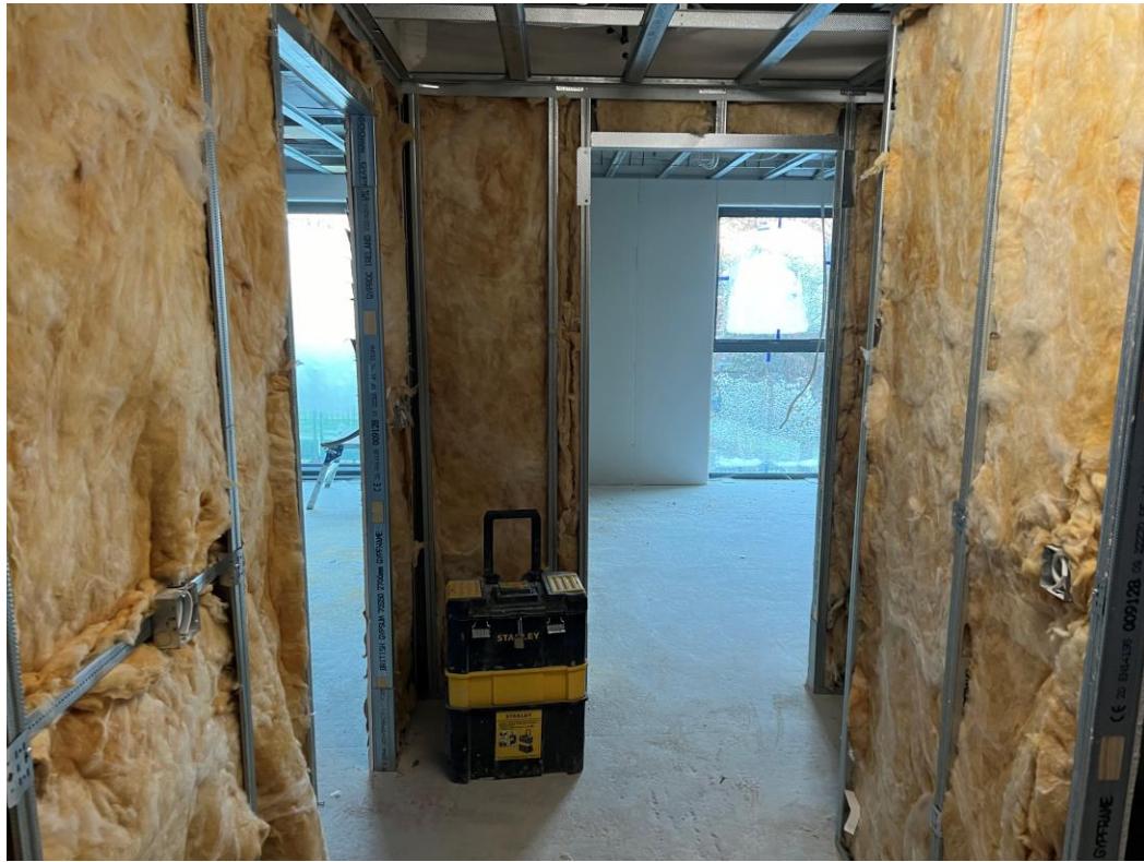
Upper levels partition wall & ceiling framework
