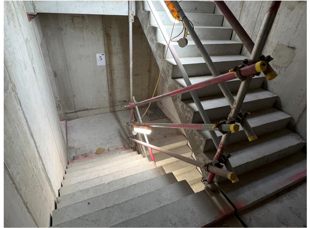
Upper floor staiwell
