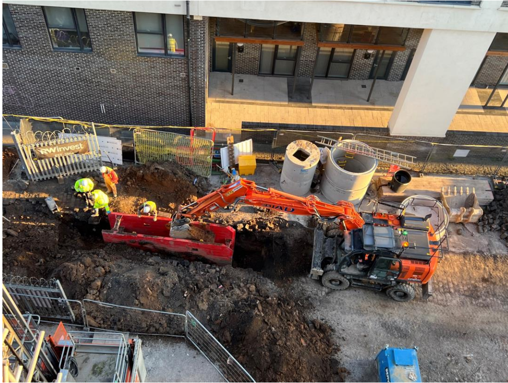
Underground drainage Dyer Street
