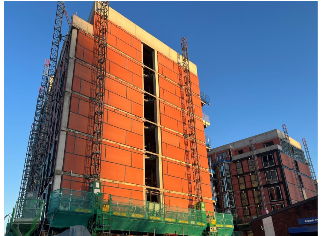
Worrall Street site view
