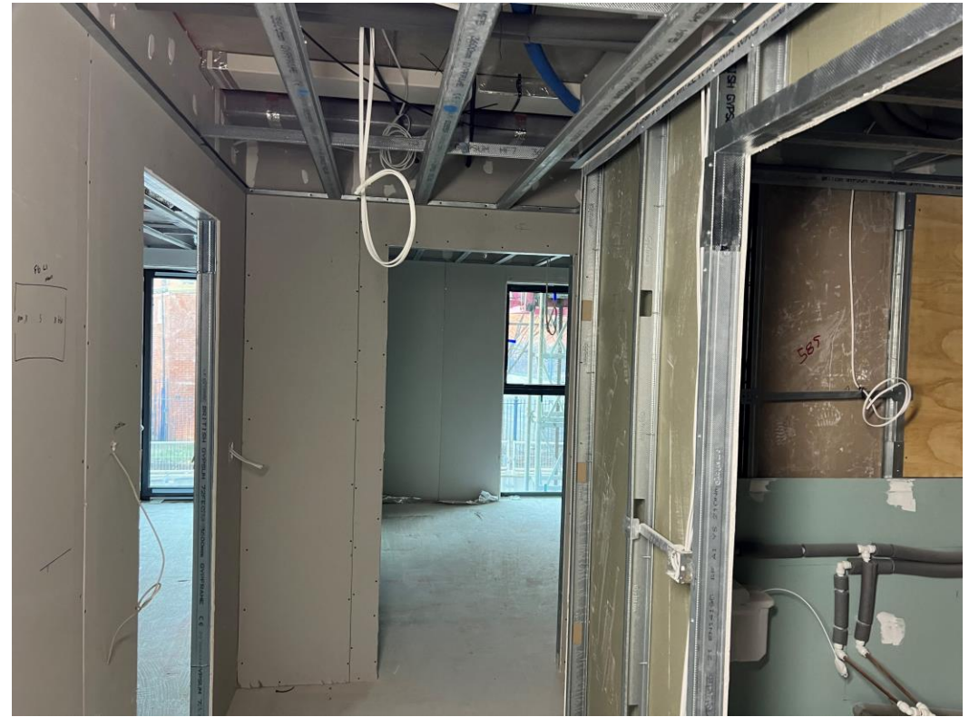
Upper levels partition wall & ceiling framework
