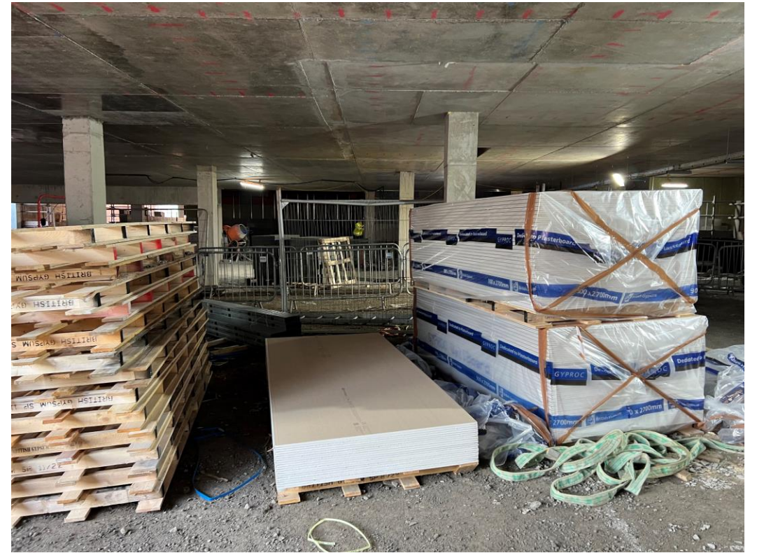
Ground floor undercroft – Material storage
