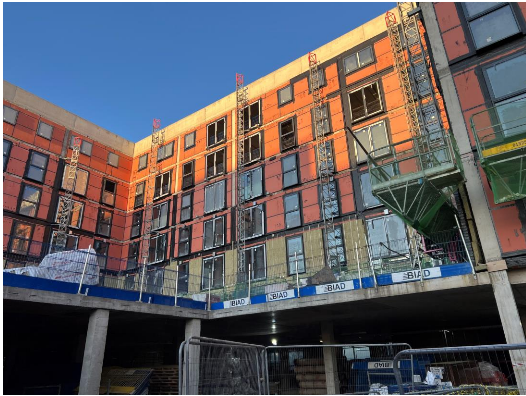
Block B – Weatherboarding, windows & doors installed
