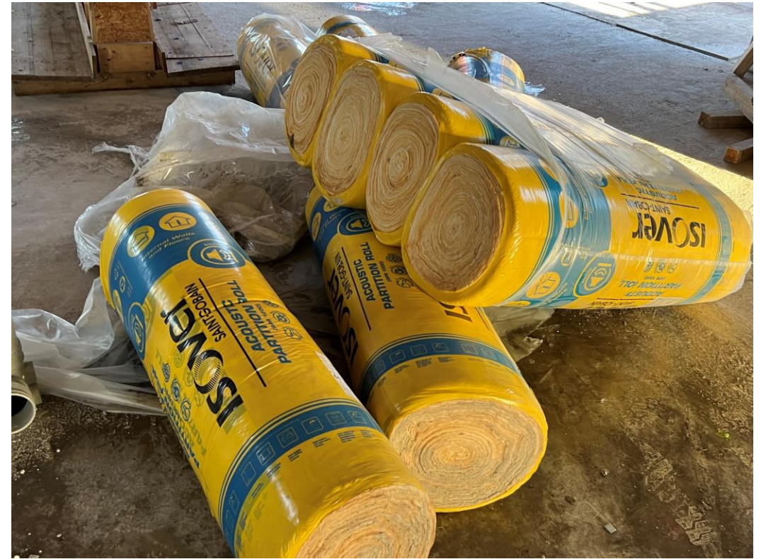
Upper levels partition wall materials
