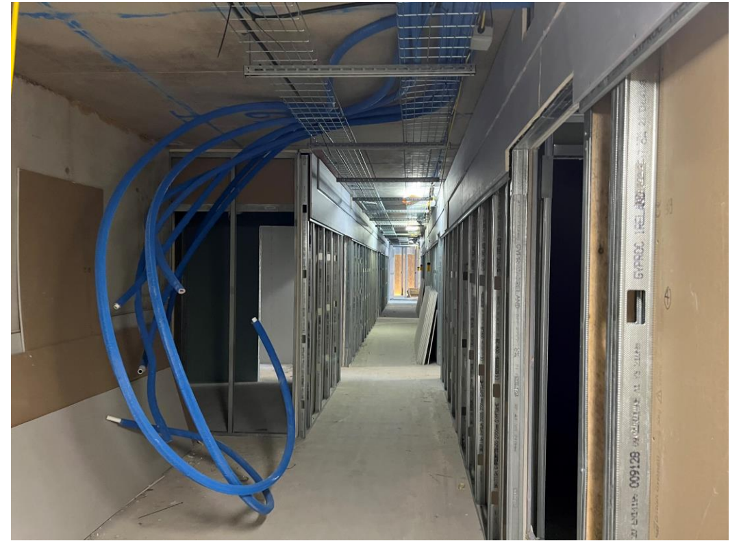
Upper level Corridor partition walls & services
