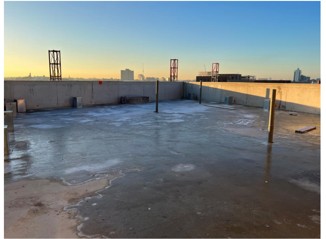
Block A – Roof Terrace
