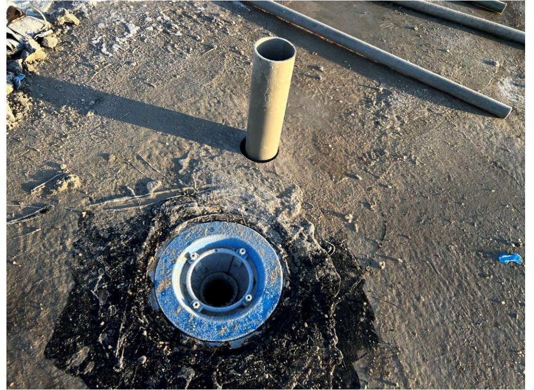
Block B – Roof outlet commenced
