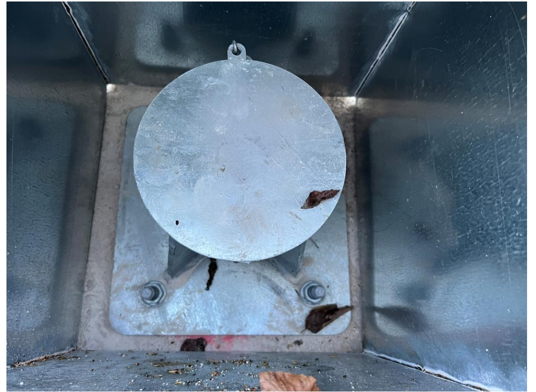
Block A – Roof drainage ventilation
