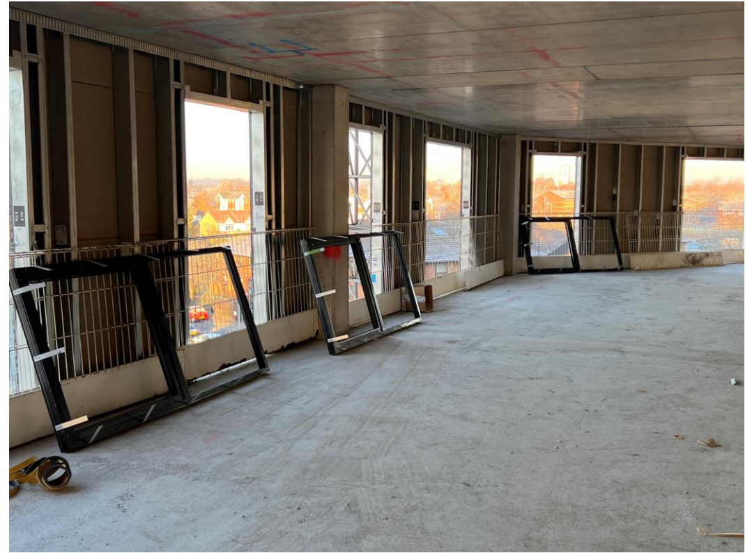
Upper level SFS and weatherboarding
