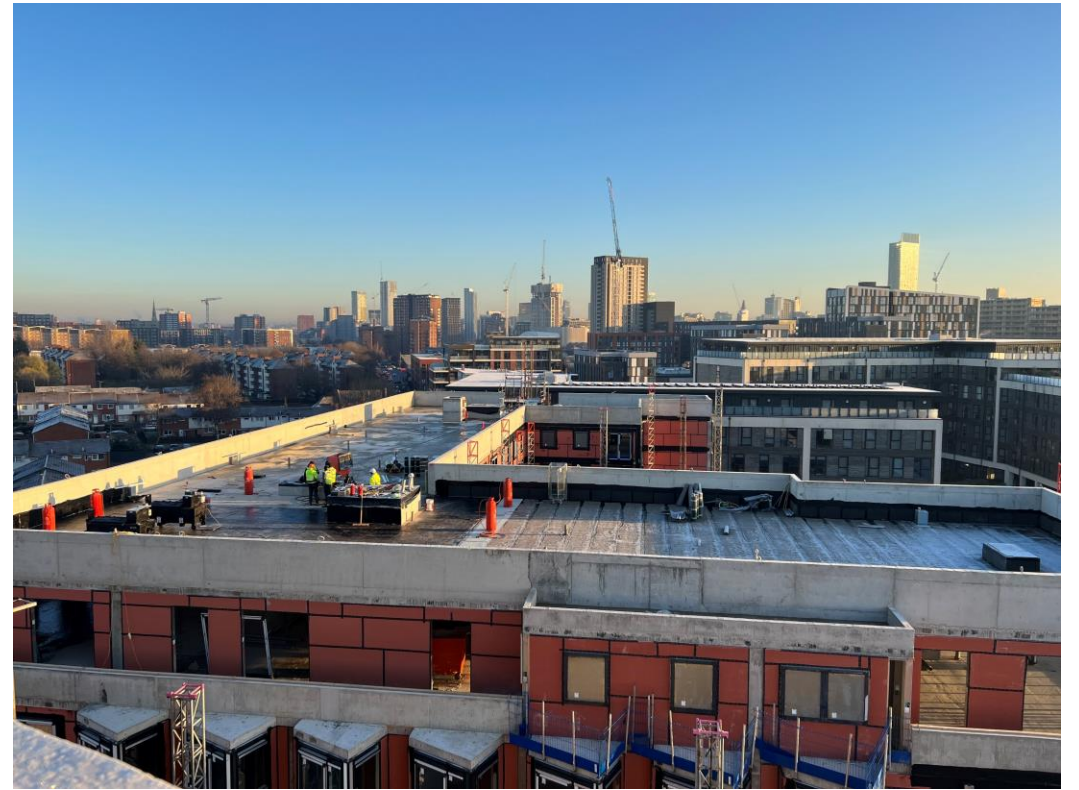
Block B roof view
