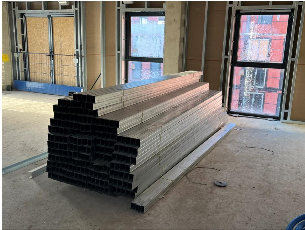
Upper levels partition wall materials
