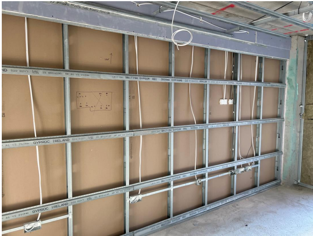
Upper levels partition wall framework
