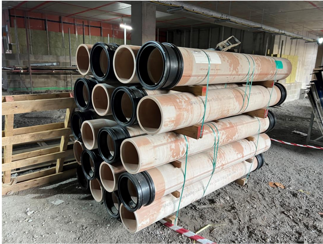
Underground drainage Dyer Street
