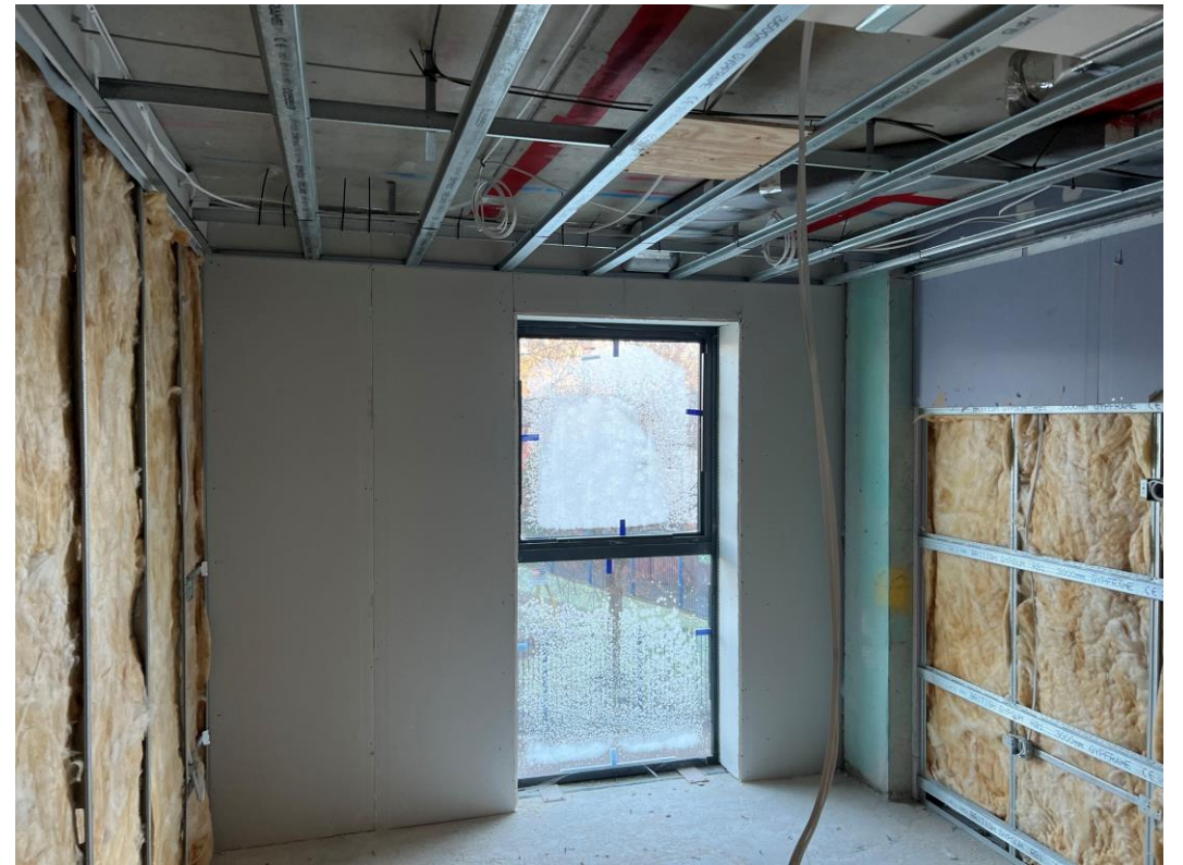
Upper levels partition wall framework
