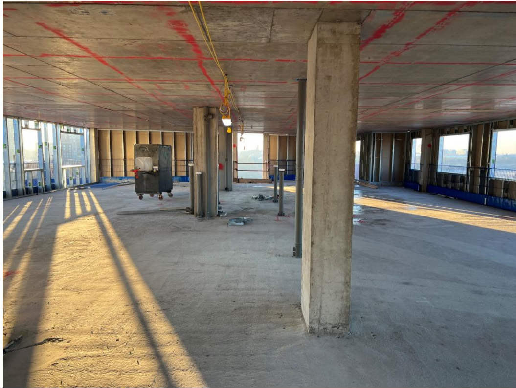
Upper level SFS and weatherboarding
