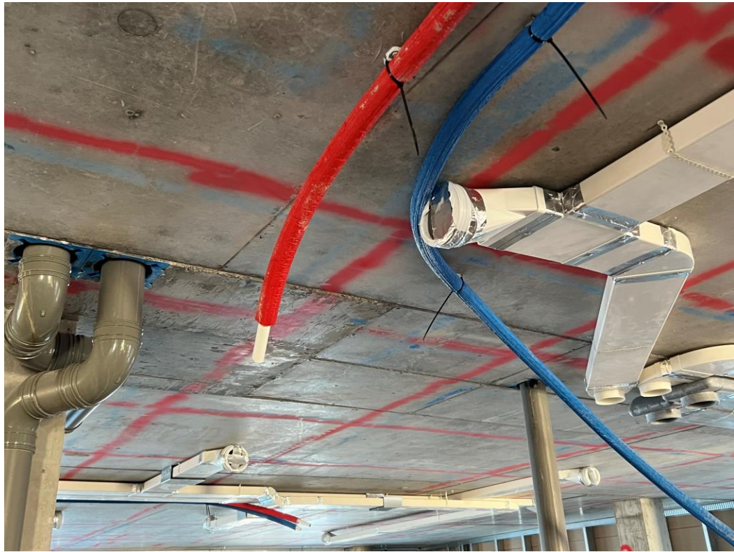
Upper levels hot and cold water supply
