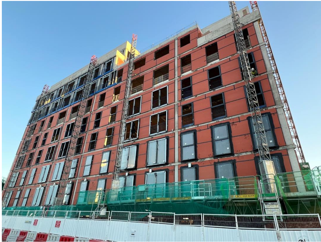
Worrall Street site view
