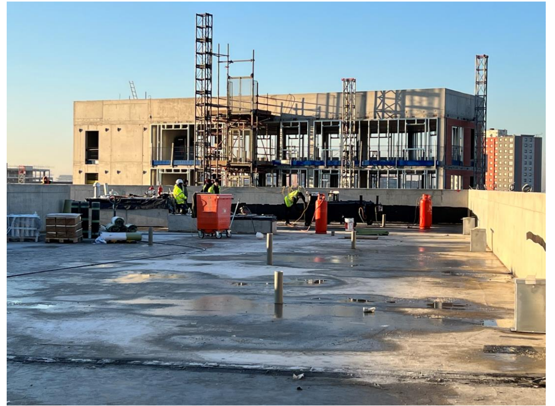
Block B – Roof covering commenced
