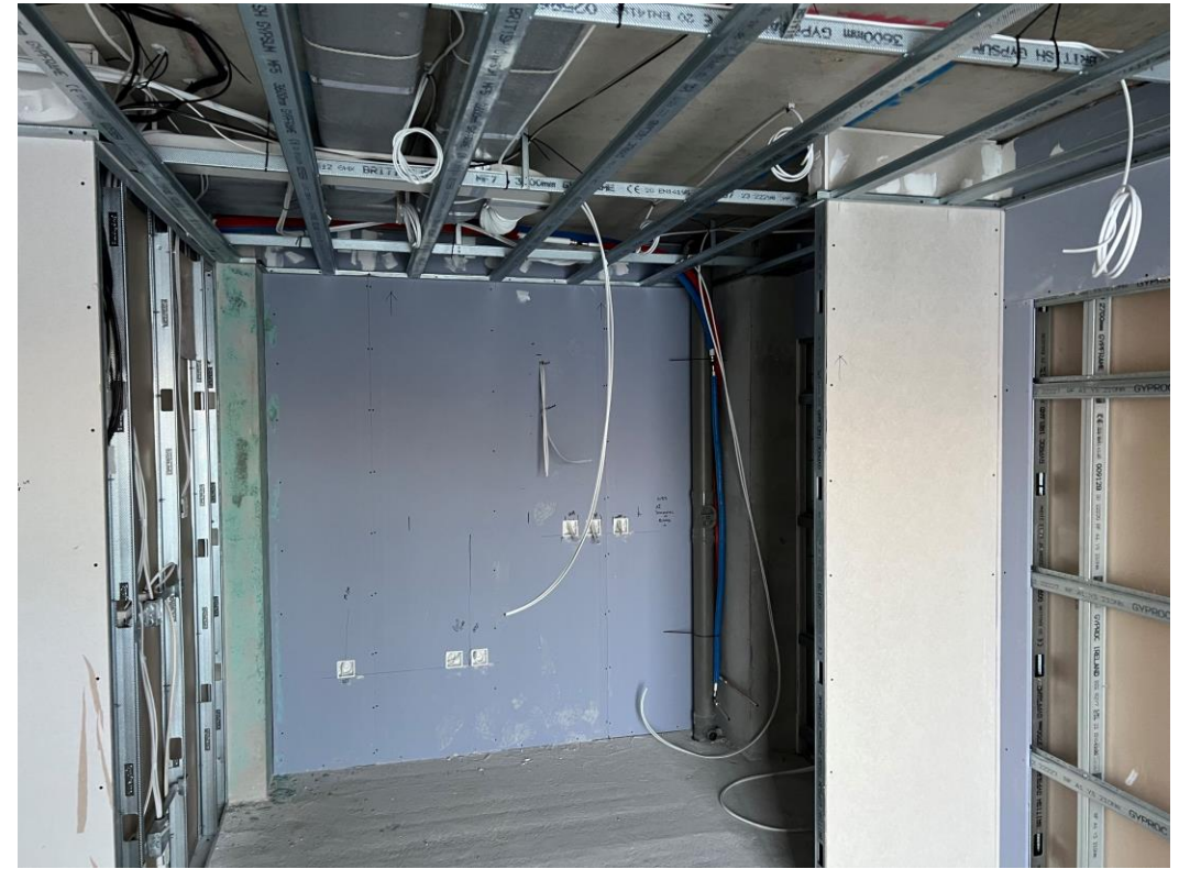
Upper level Apartment 1 st fix mechanical and electrical
