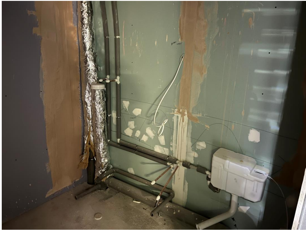
Upper level Apartment 1 st fix sanitary
