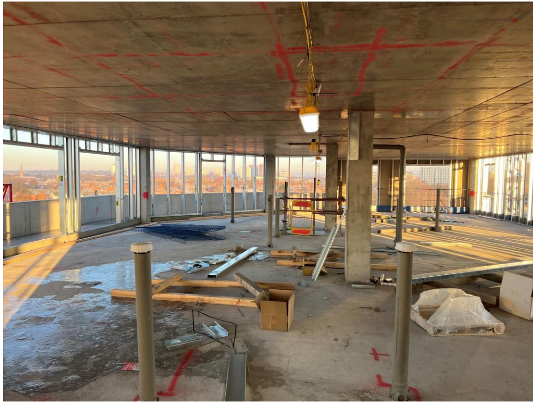
Upper level SFS external walls
