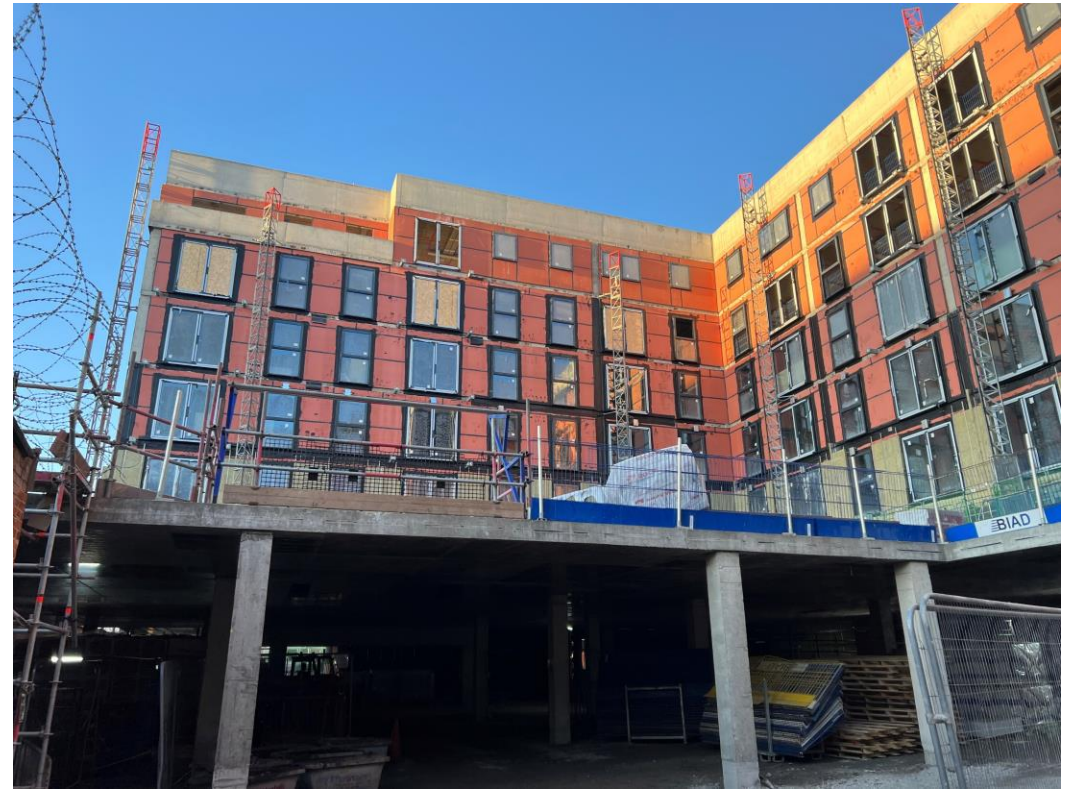
Block B – Weatherboarding, windows & doors installed
