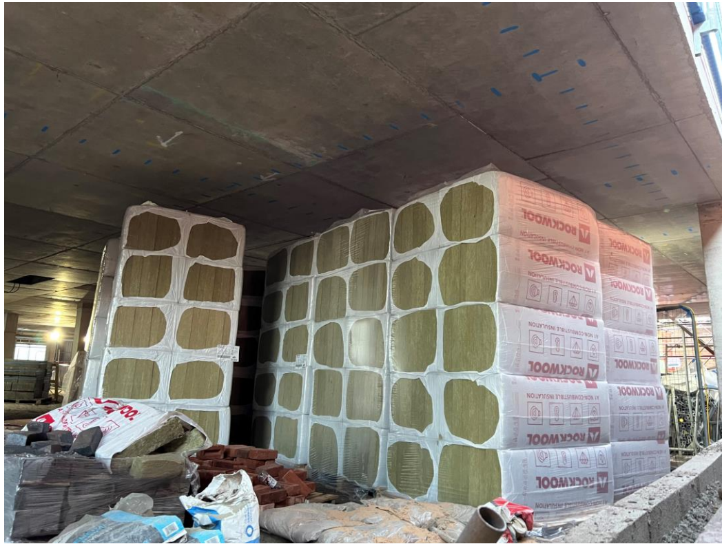
Ground floor undercroft – Material storage
