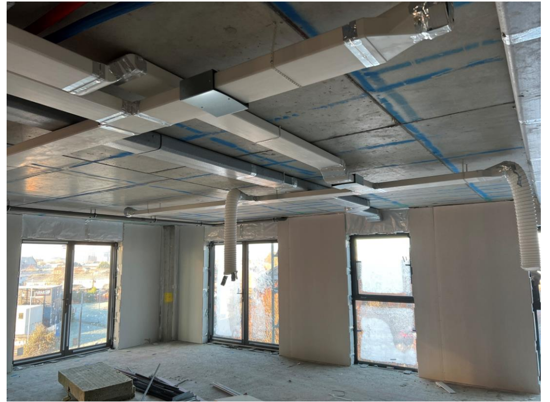
Upper level Apartment 1 st fix mechanical
