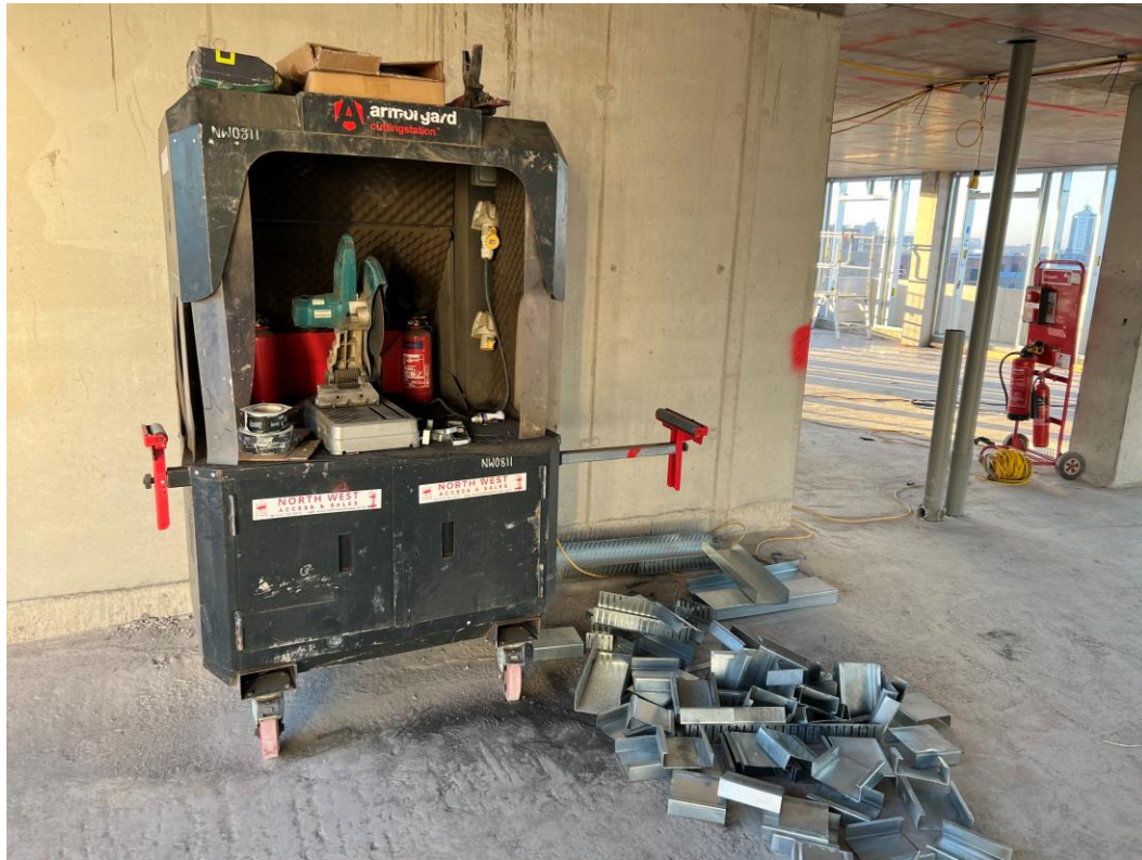
Upper level SFS installation
