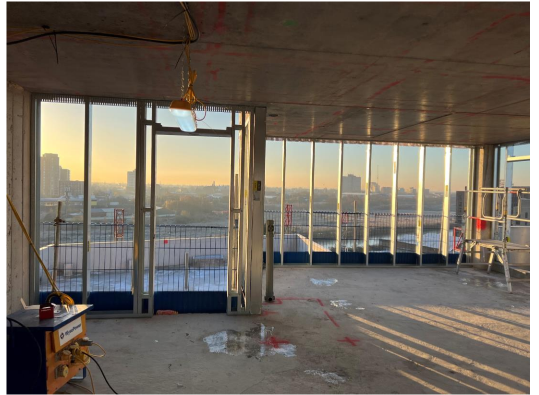
Upper level SFS external walls
