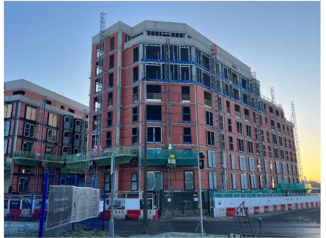
Ordsall Lane site view
