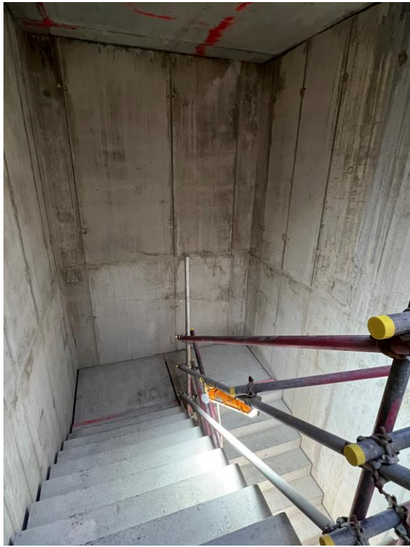
Upper floor staiwell
