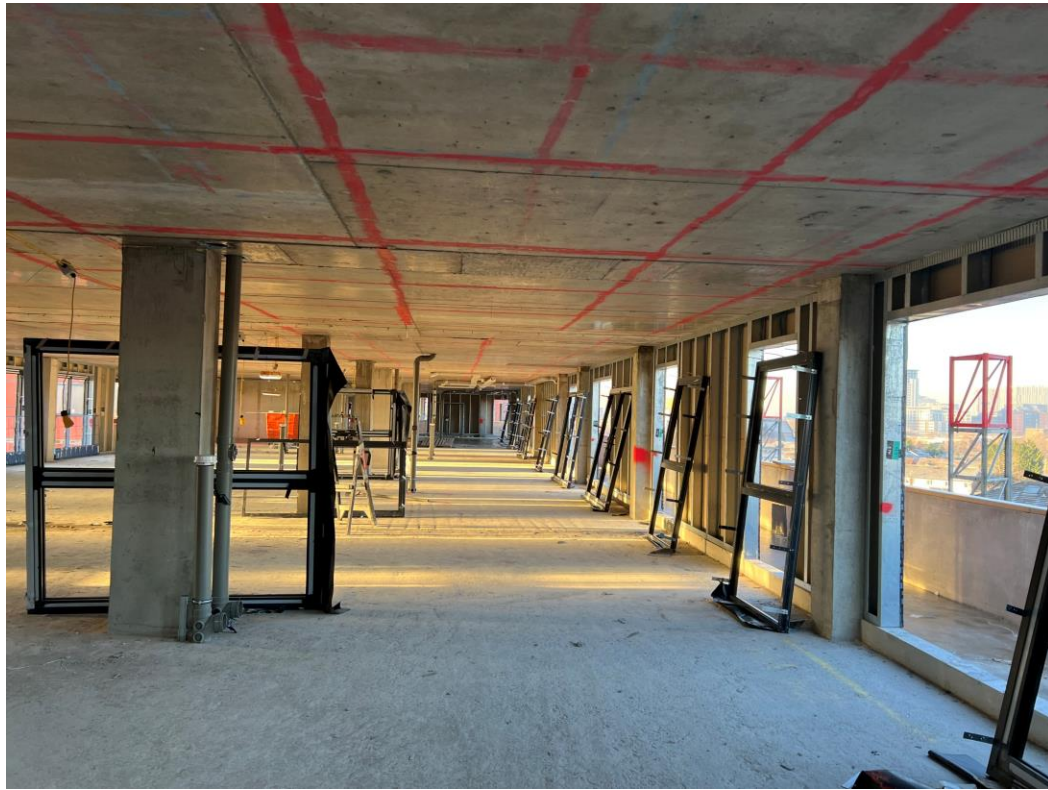
Upper levels windows installation
