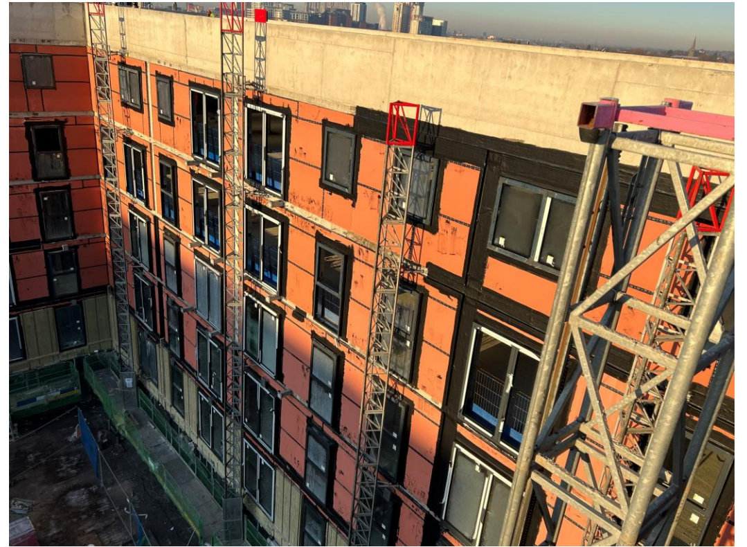
Block B – Weatherboarding, windows & doors installed
