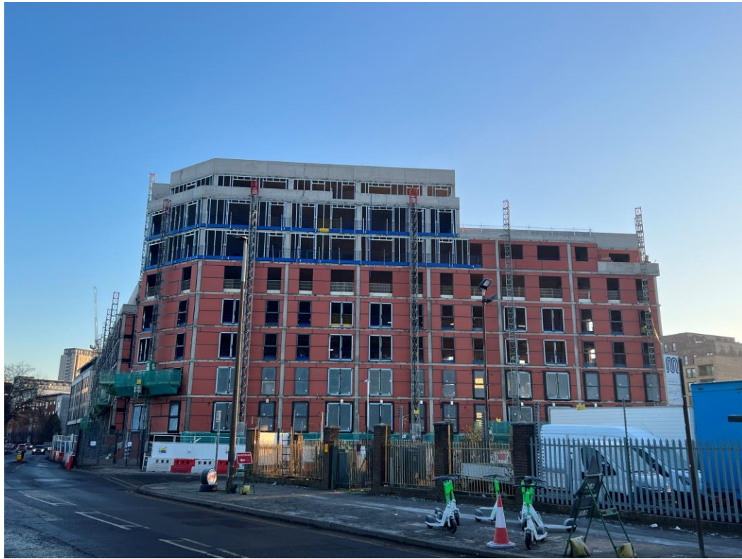
Ordsall Lane site view
