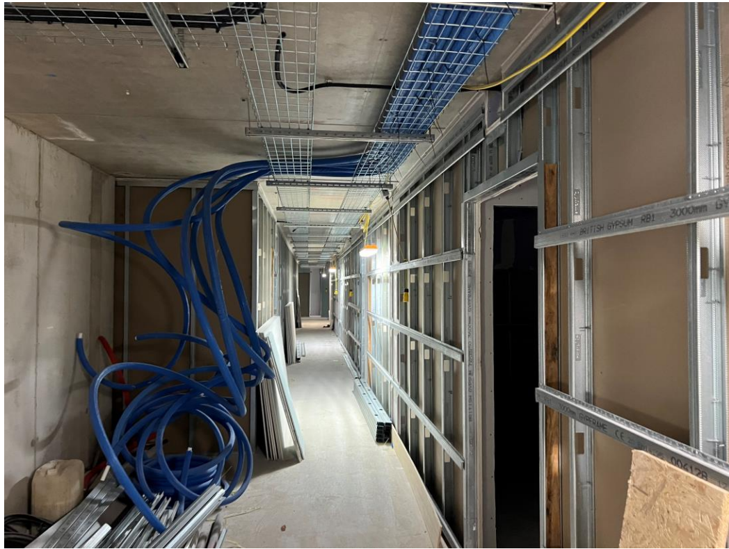
Upper level Corridor partition walls & services
