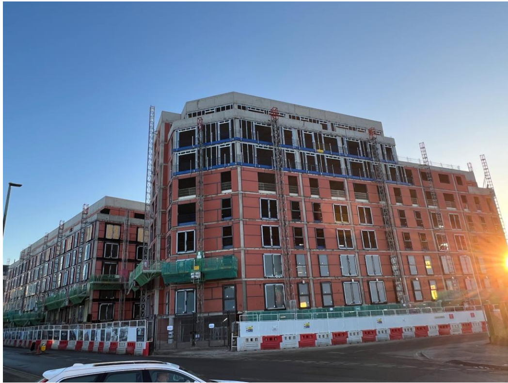
Ordsall Lane site view
