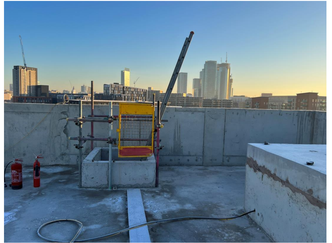
Block B – Roof outlet commenced
