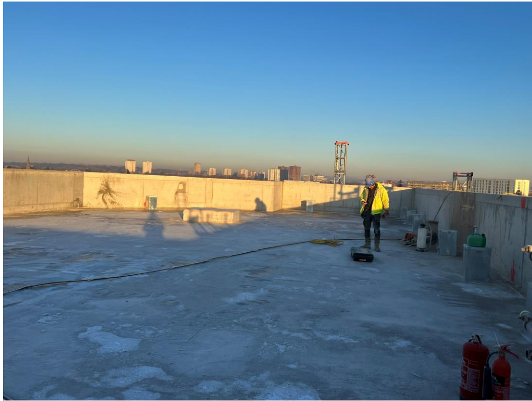
Block A – Roof covering preparation
