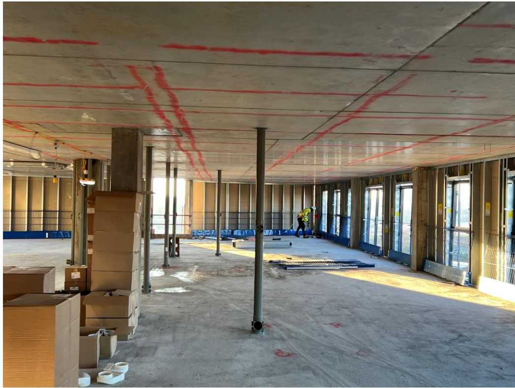
Upper level windows installed
