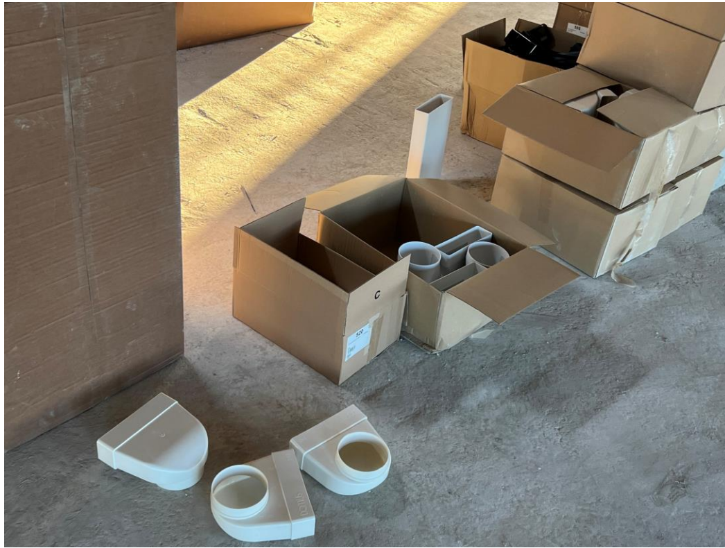
Upper level 1 st fix mechanical ducting
