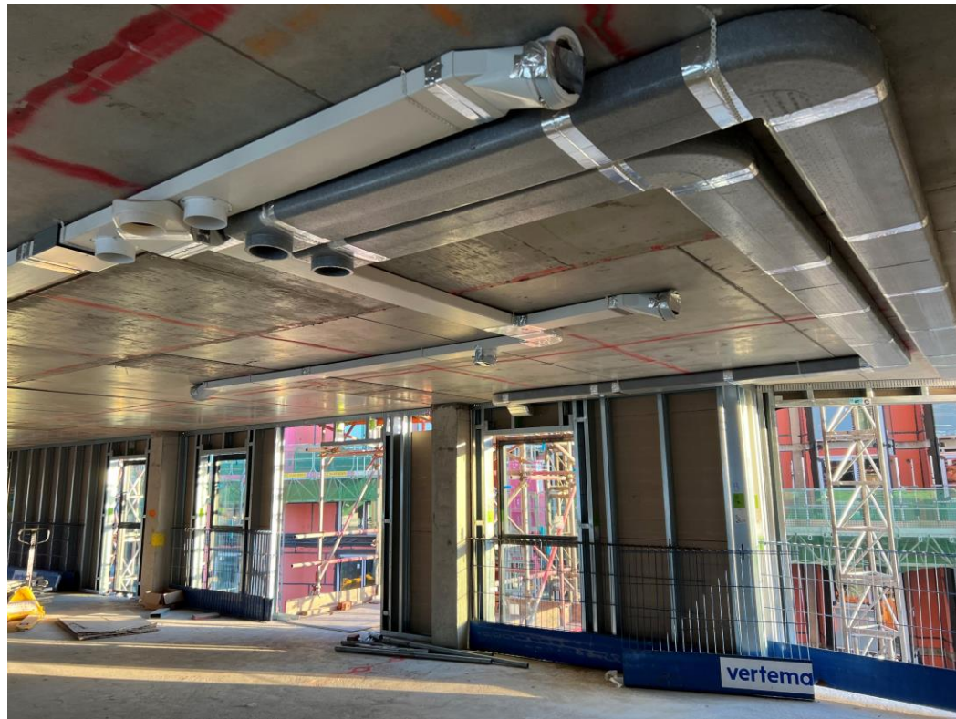
Upper level 1 st fix mechanical ducting
