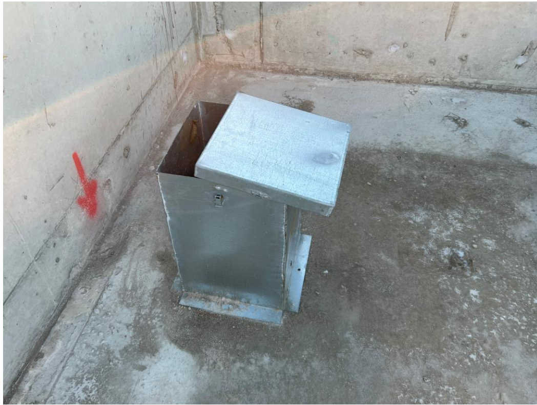
Block A – Roof drainage ventilation
