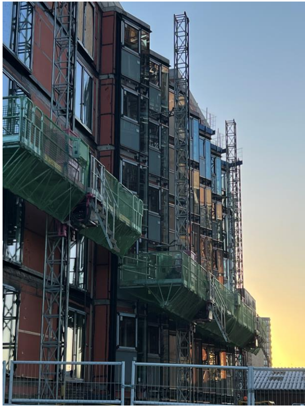
Ordsall Lane site view
