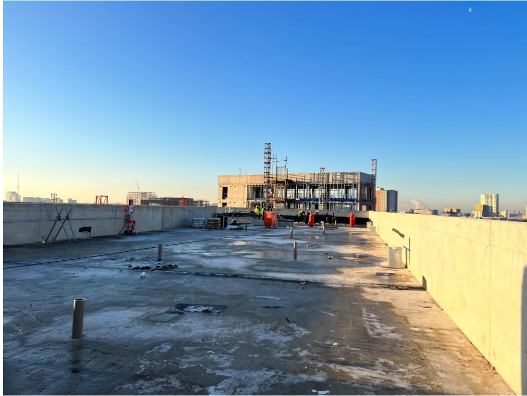
Block B – Roof covering commenced
