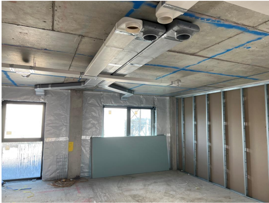
Upper level Apartment 1 st fix mechanical
