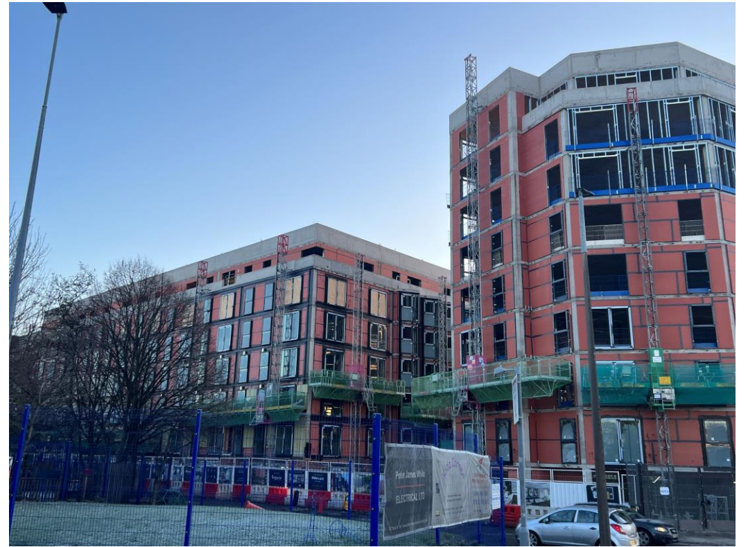
Ordsall Lane site view
