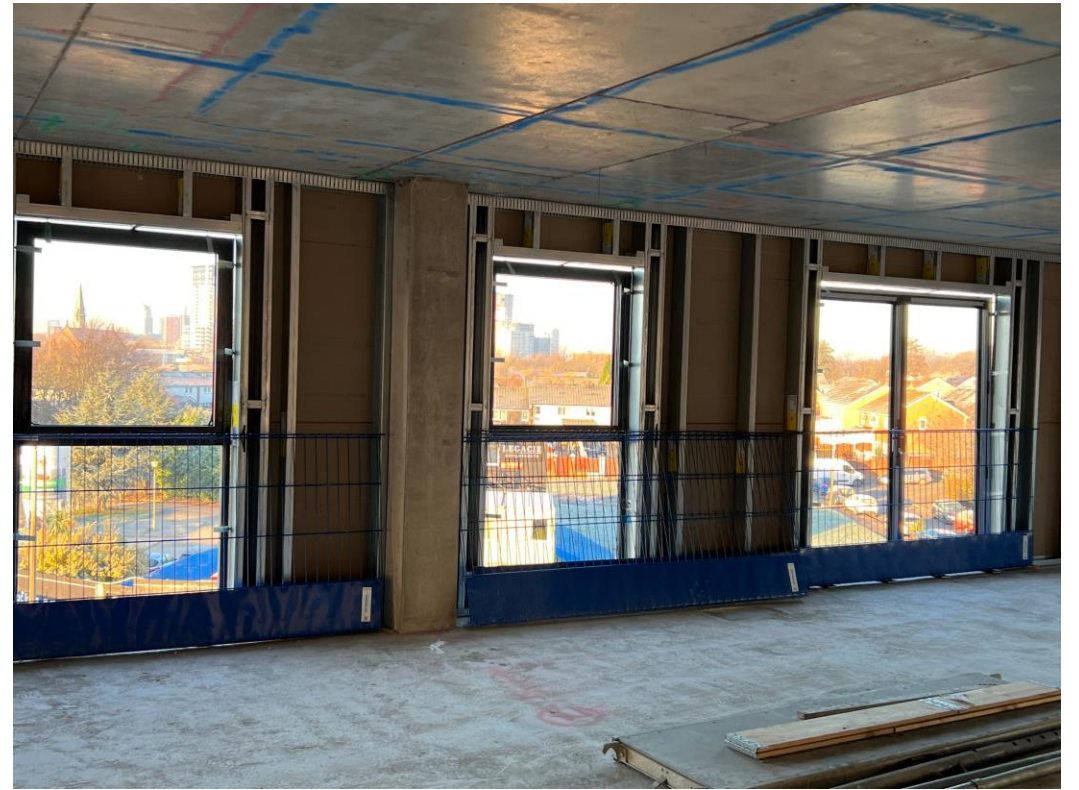
Upper level windows installed
