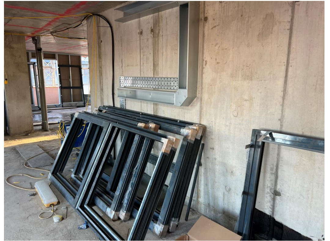
Upper levels windows installation
