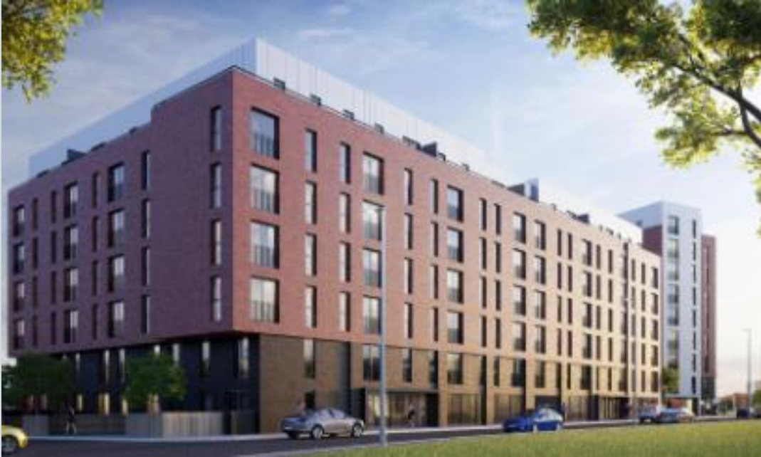
Land at corner of Ordsall Lane, Dyer Street & Worrall Street, Salford, Manchester M5
