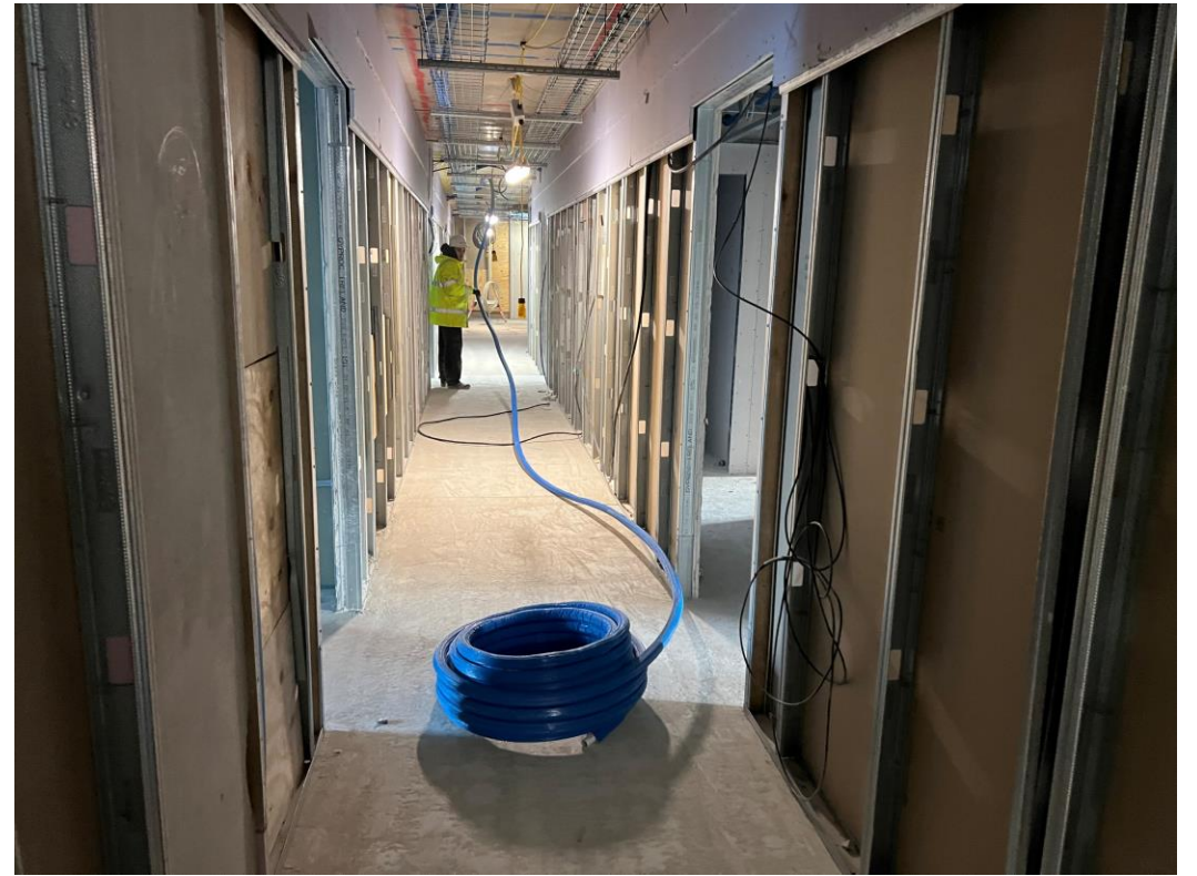
Upper level Corridor partition walls & services
