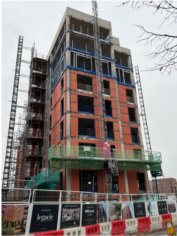
Ordsall Lane site view
