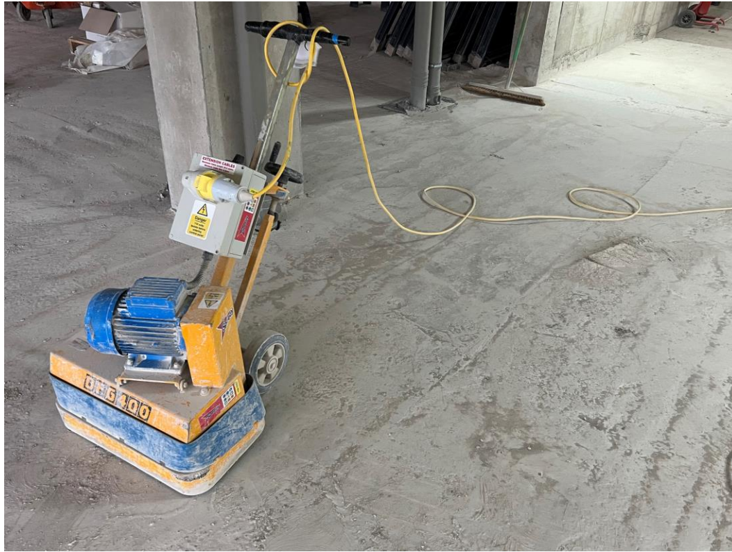
Upper level floor slab preparation
