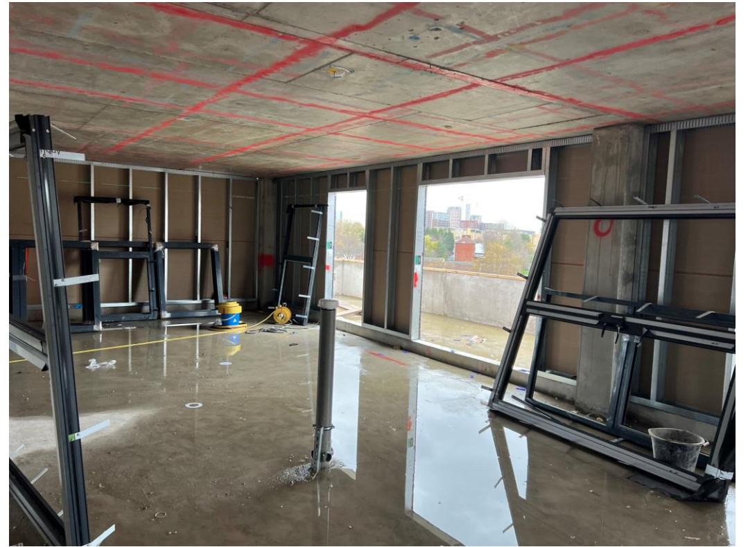
Upper levels SFS and weatherboarding, windows to install
