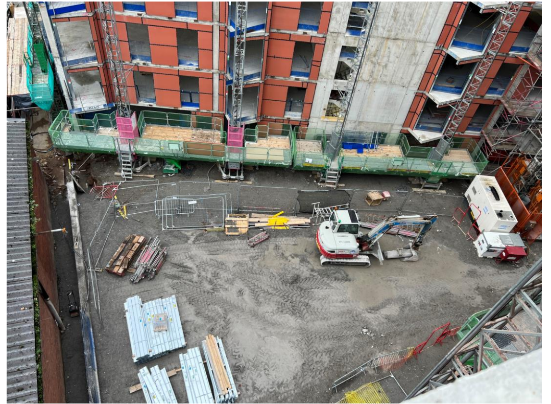
Block A – SFS & weatherboarding installed
