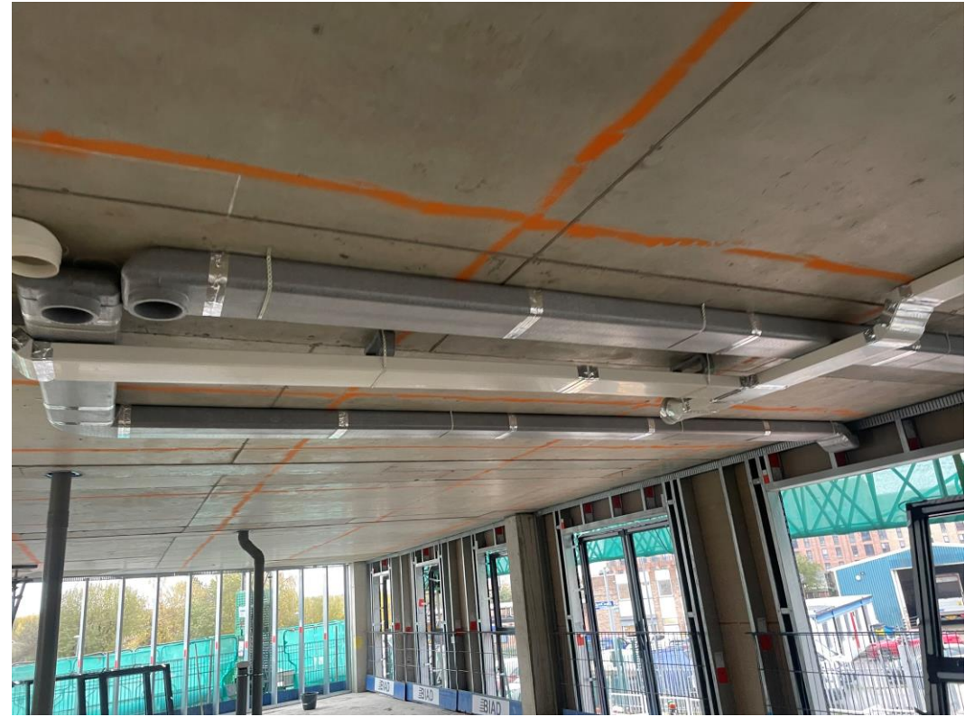
First floor 1 st fix mechanical ducting
