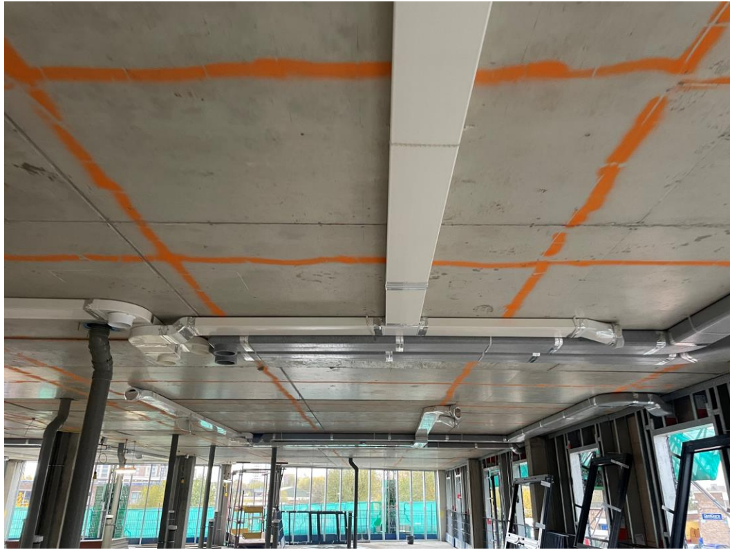
First floor 1 st fix mechanical ducting
