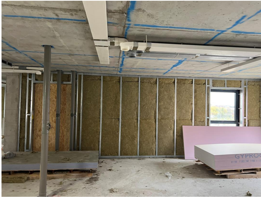
Upper levels insulation external walls
