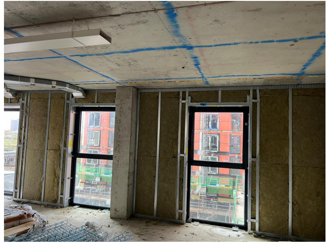
Upper levels insulation external walls
