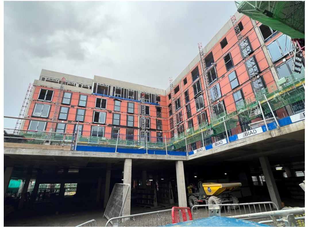
Block B – Podium complete
