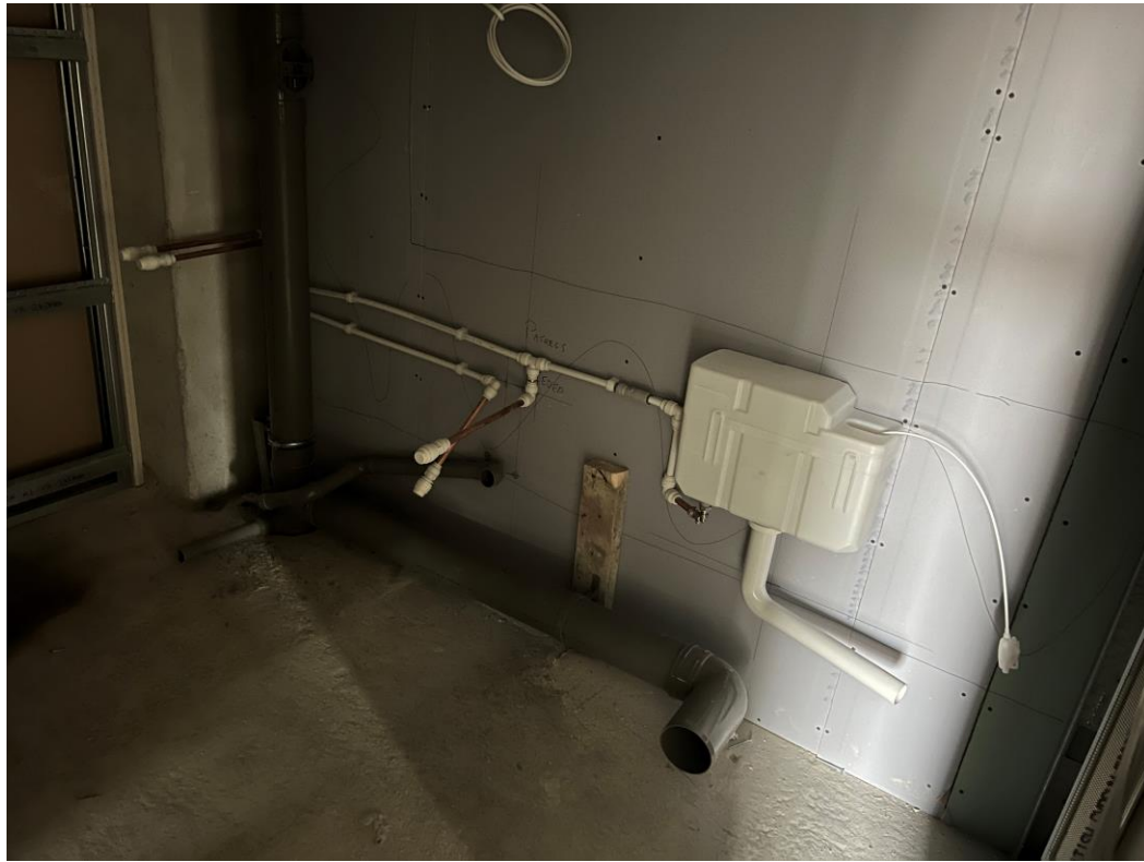
Upper level Apartment 1 st fix sanitary
