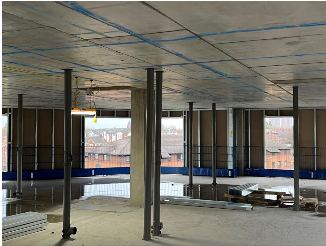
Upper level SFS and weatherboarding
