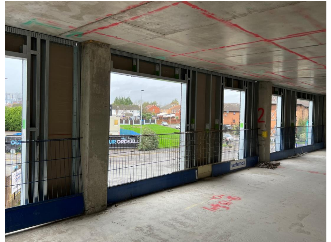
Upper level SFS and weatherboarding
