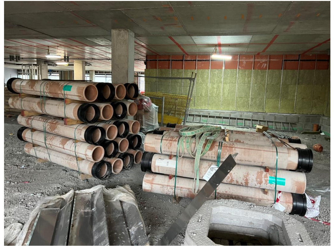
Ground floor undercroft
