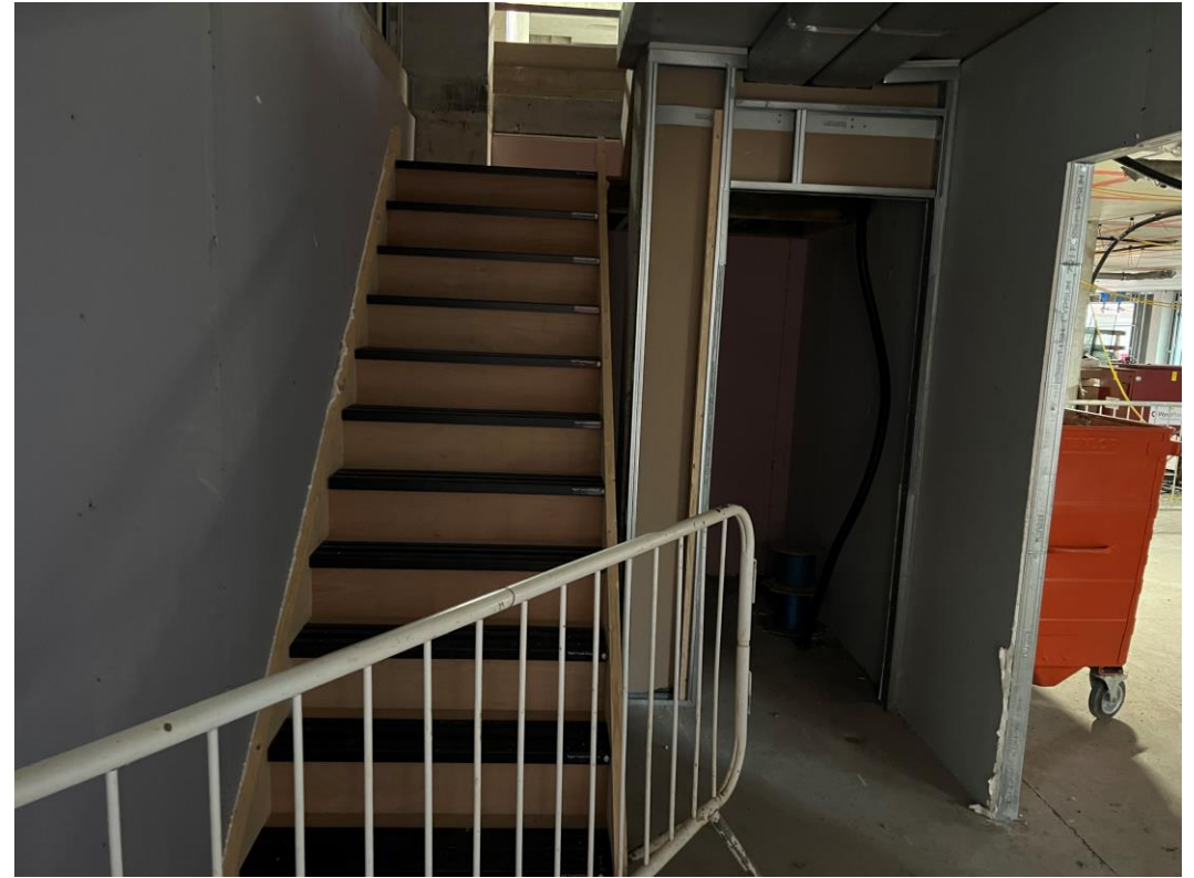
Ground floor partition walls & staircase
