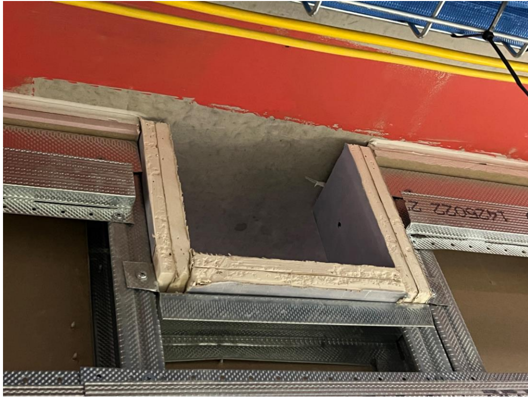
Upper level Corridor partition walls & services
