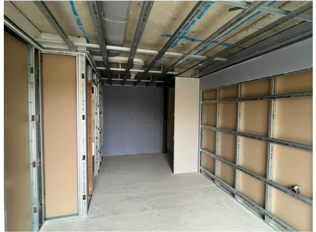
Upper level Apartment partition walls & ceiling formed
