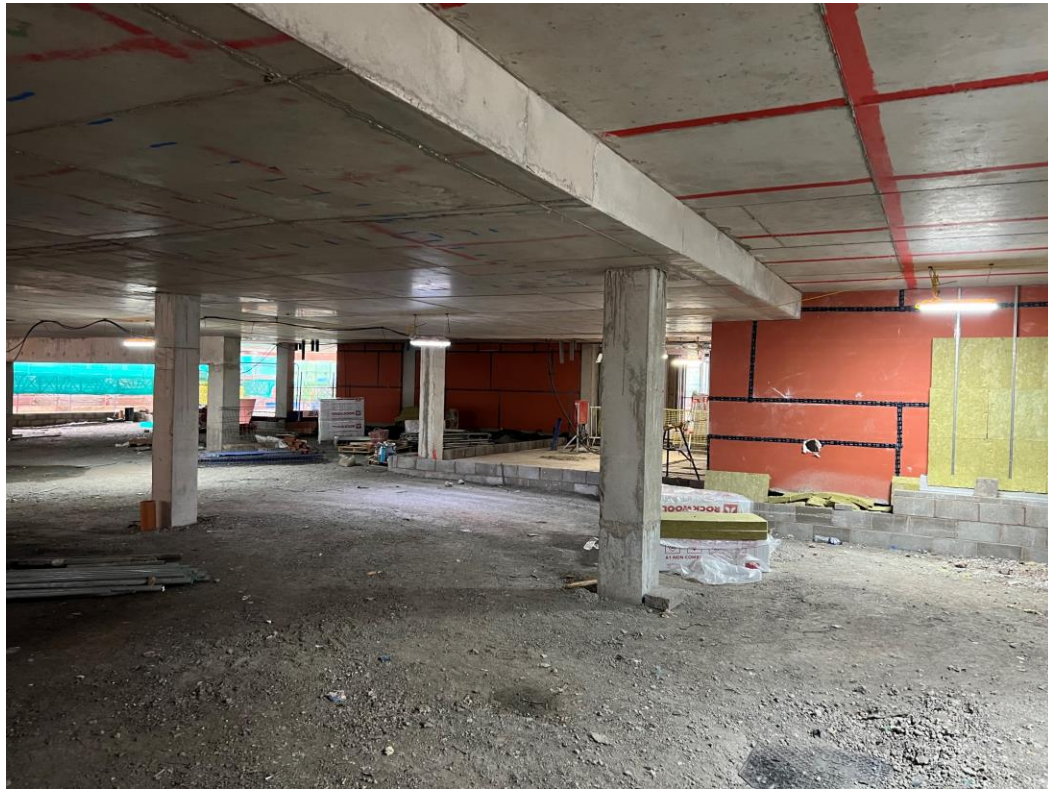
Ground floor undercroft
