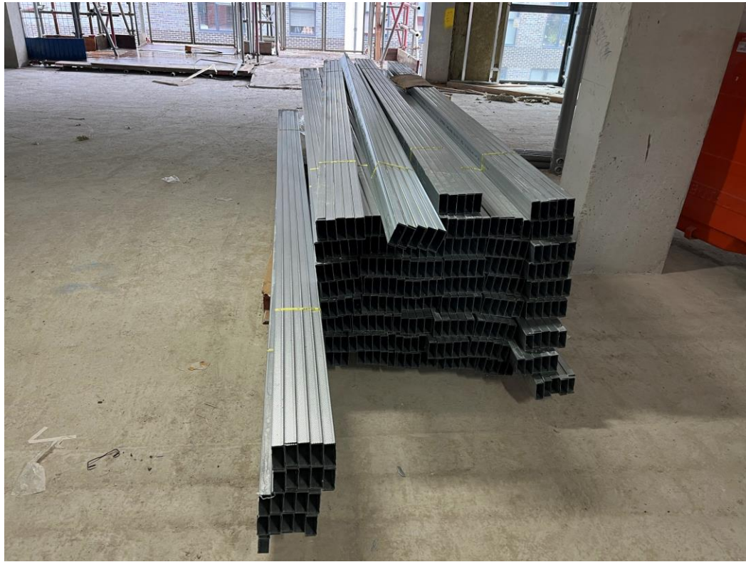
Upper levels partition wall materials
