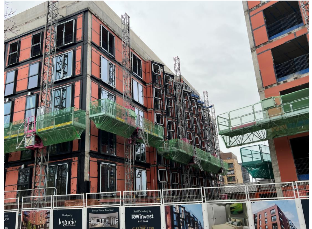
Ordsall Lane site view
