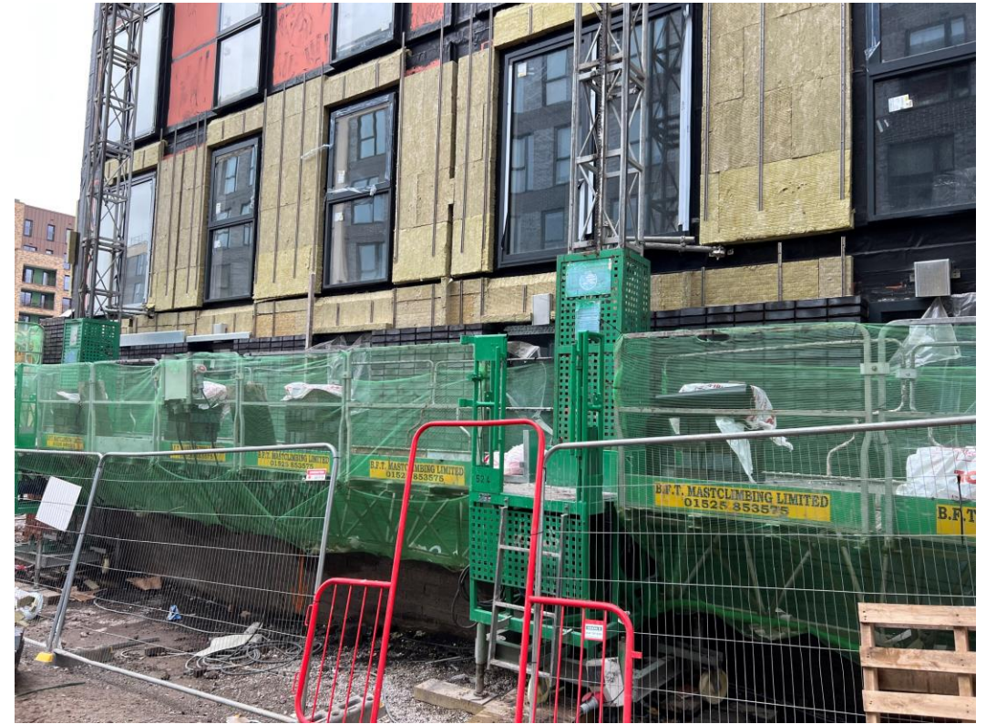
Block B – External brickwork construction
