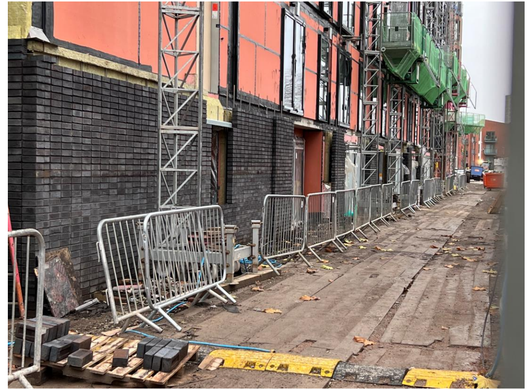
Block B – External brickwork construction
