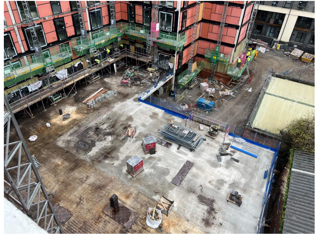
Block B – Podium complete
