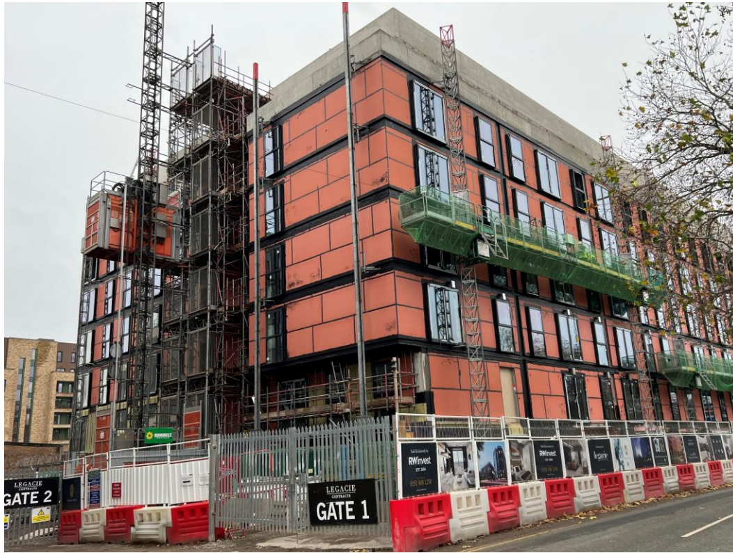
Ordsall Lane site view
