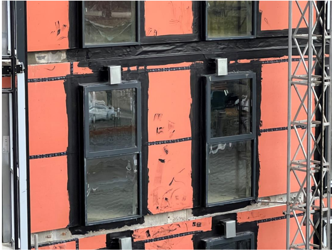
Block B – Vents installed
