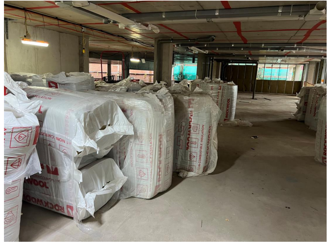
Ground floor undercroft
