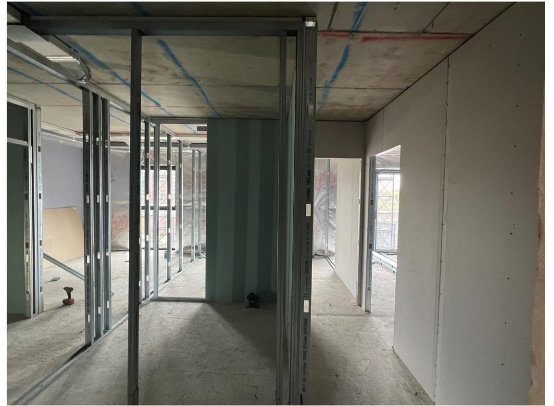
Upper levels partition wall framework
