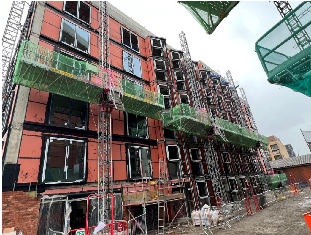
Block B – Weatherboarding, windows & doors installed
