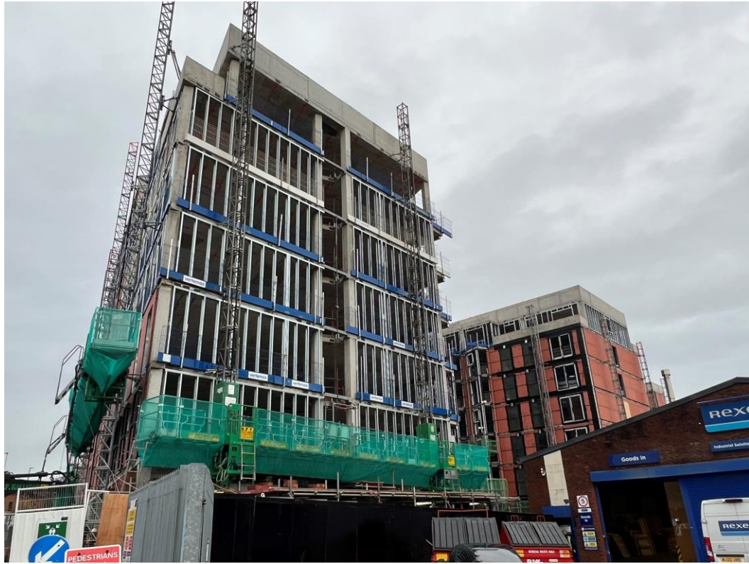
Worrall Street site view
