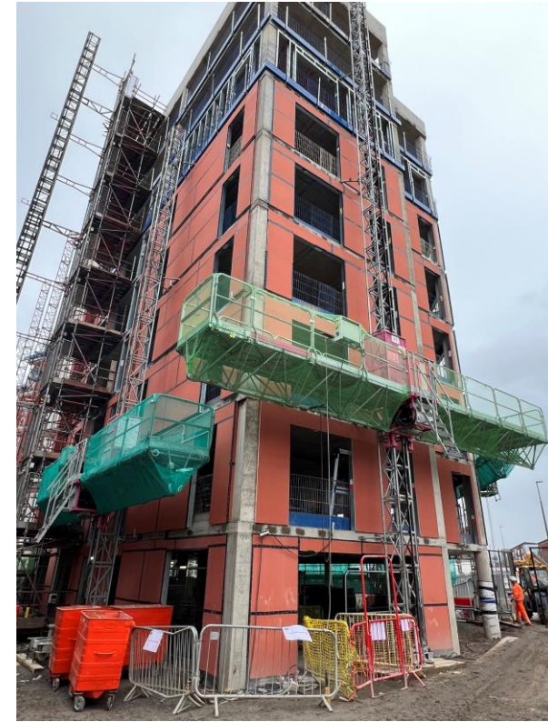
Block B – Weatherboarding, windows & doors installed
