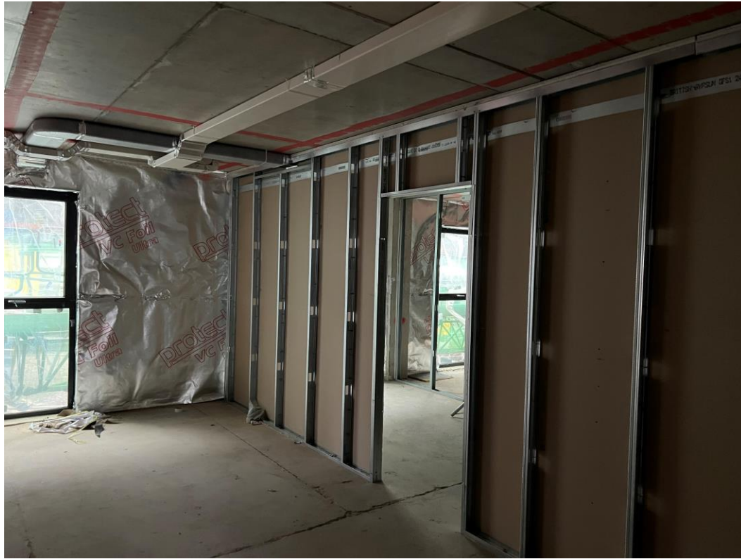
Ground floor partition walls & VCL external
