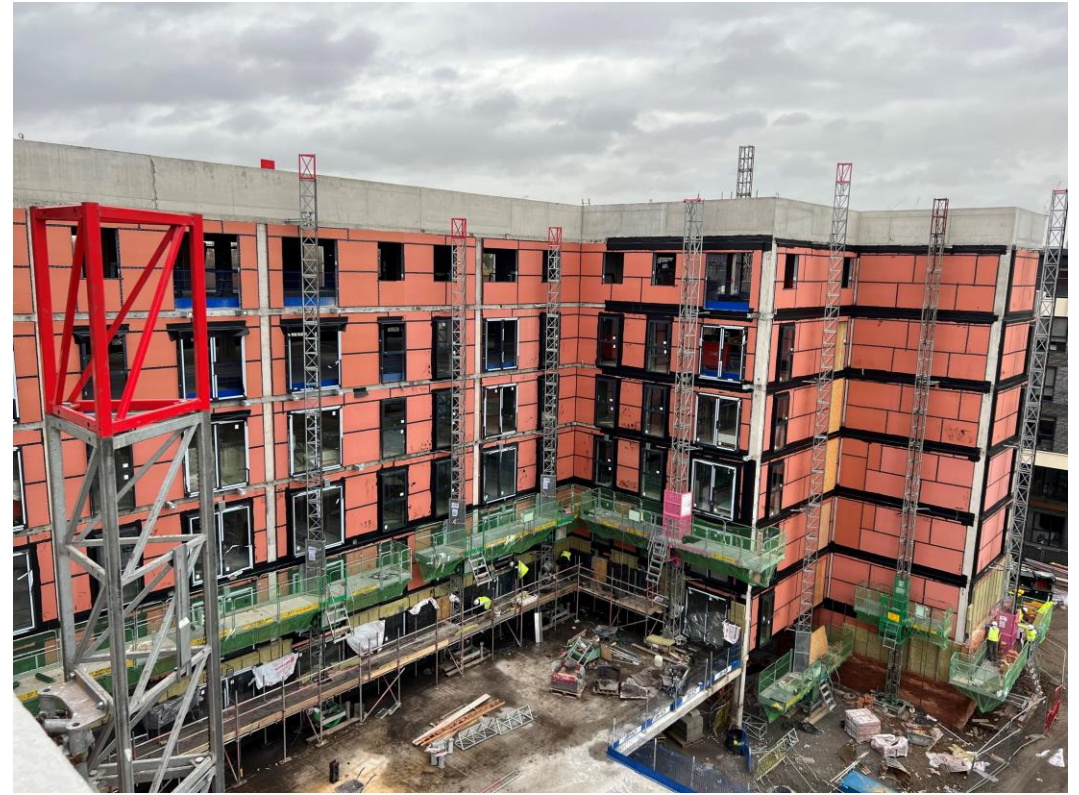
Block B – Weatherboarding, windows & doors installed
