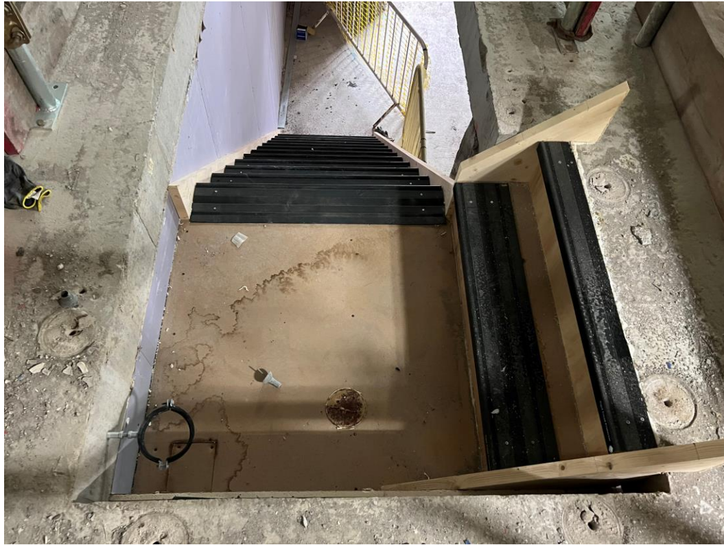
Upper levels timber staircase
