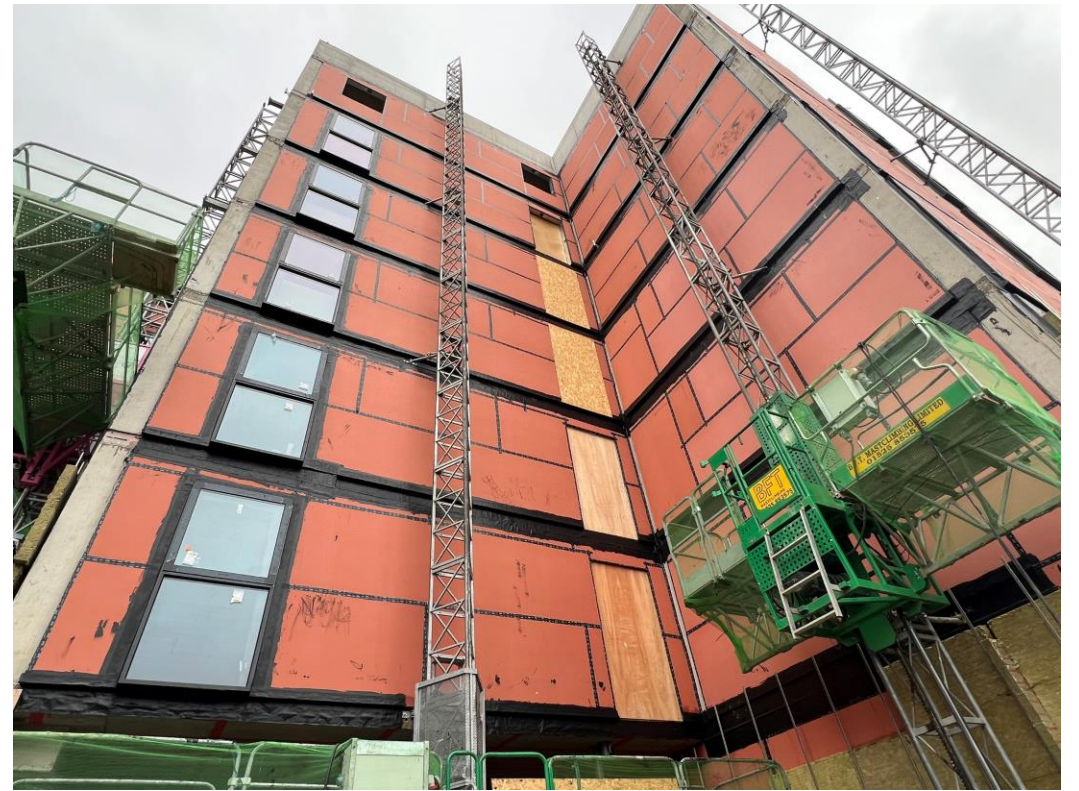
Block B – Weatherboarding, windows & doors installed
