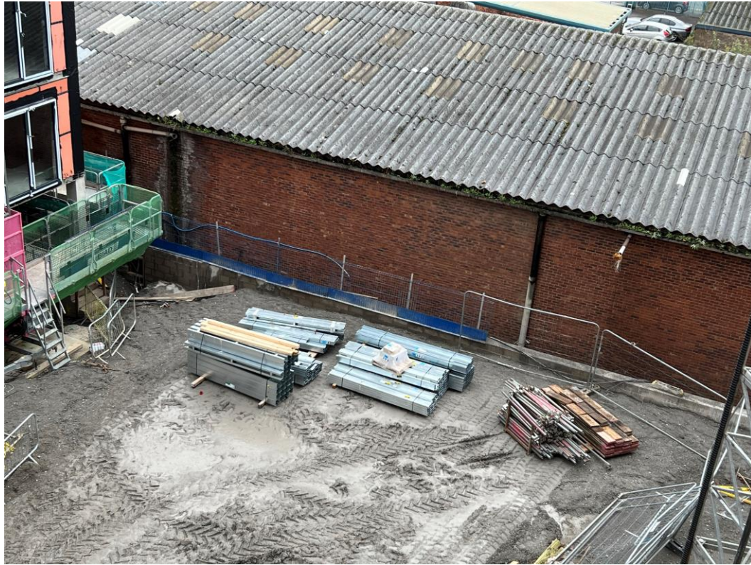
Block B – Retaining wall structure
