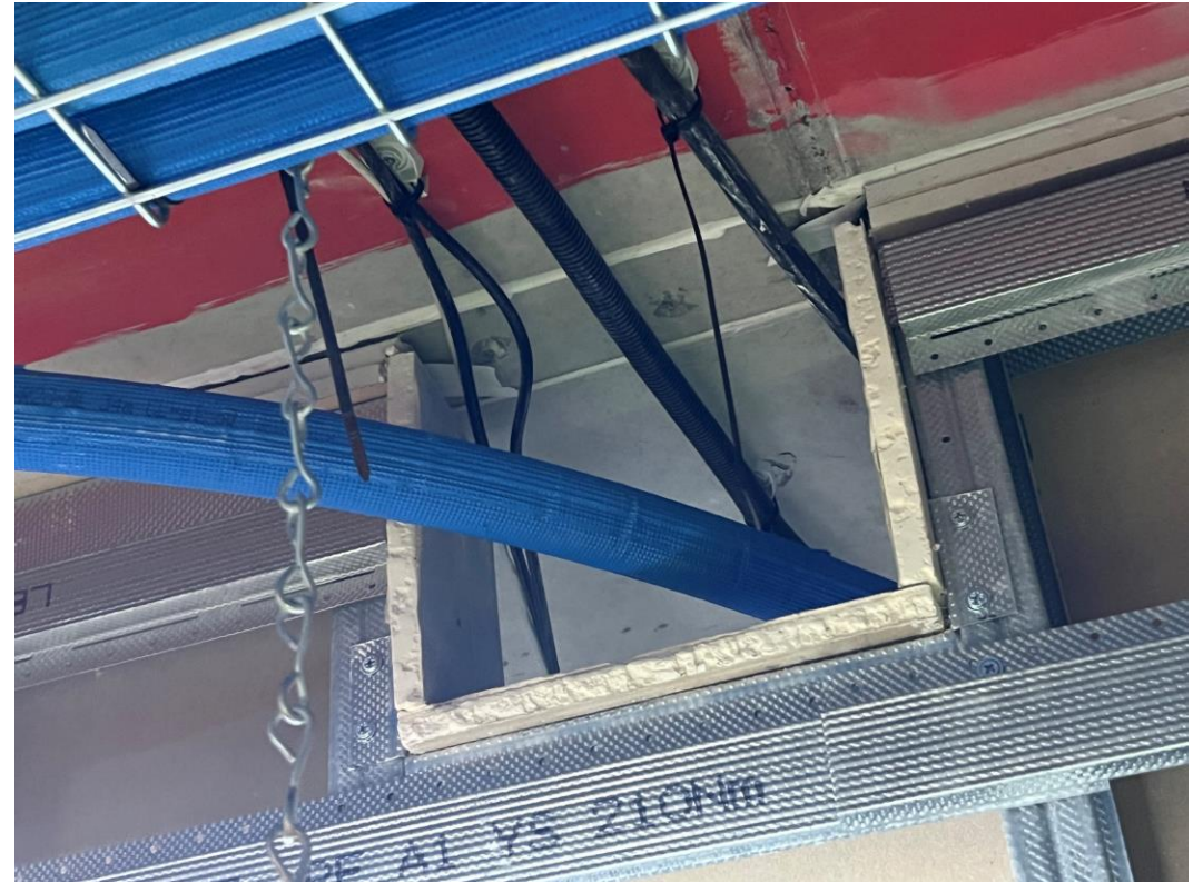
Upper level Corridor partition walls & services
