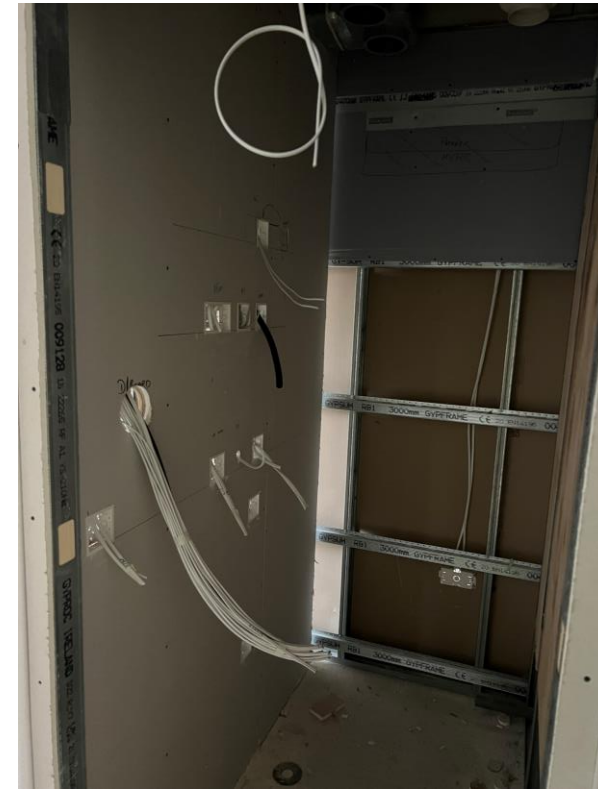
Upper level Apartment 1 st fix mechanical and electrical
