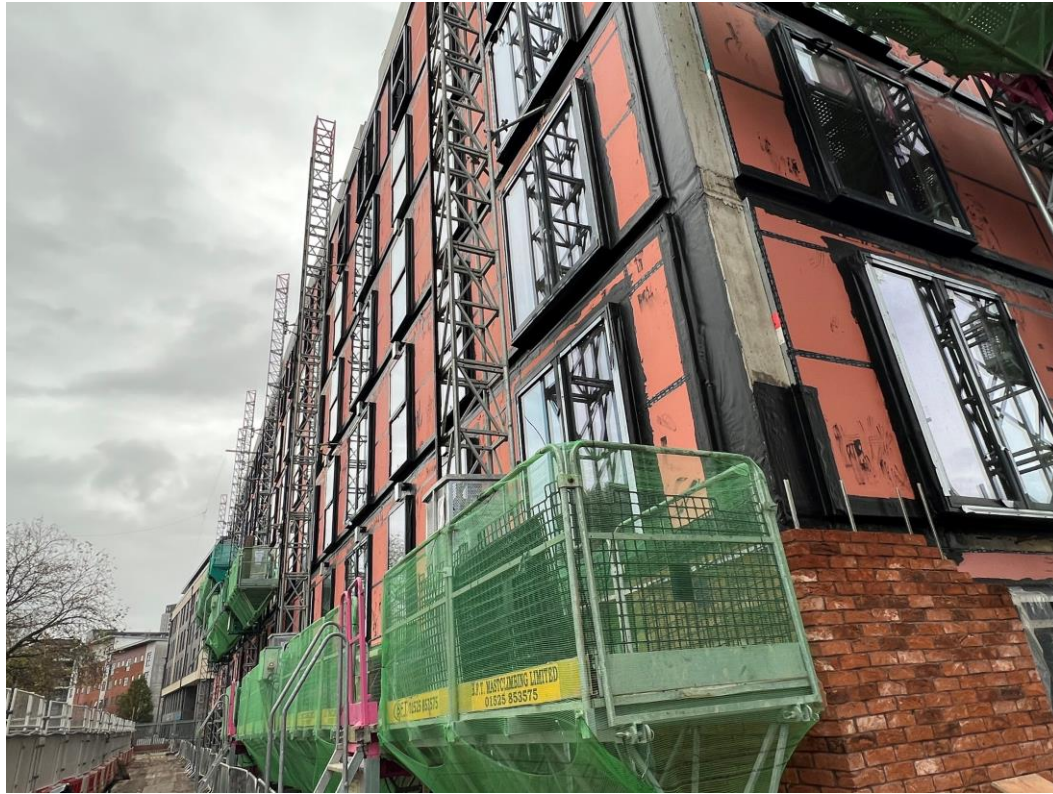
Block B – Weatherboarding, windows & doors installed
