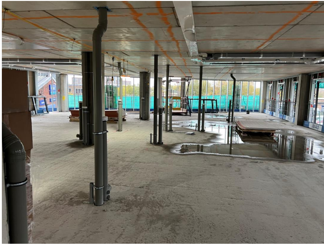
First floor above ground drainage
