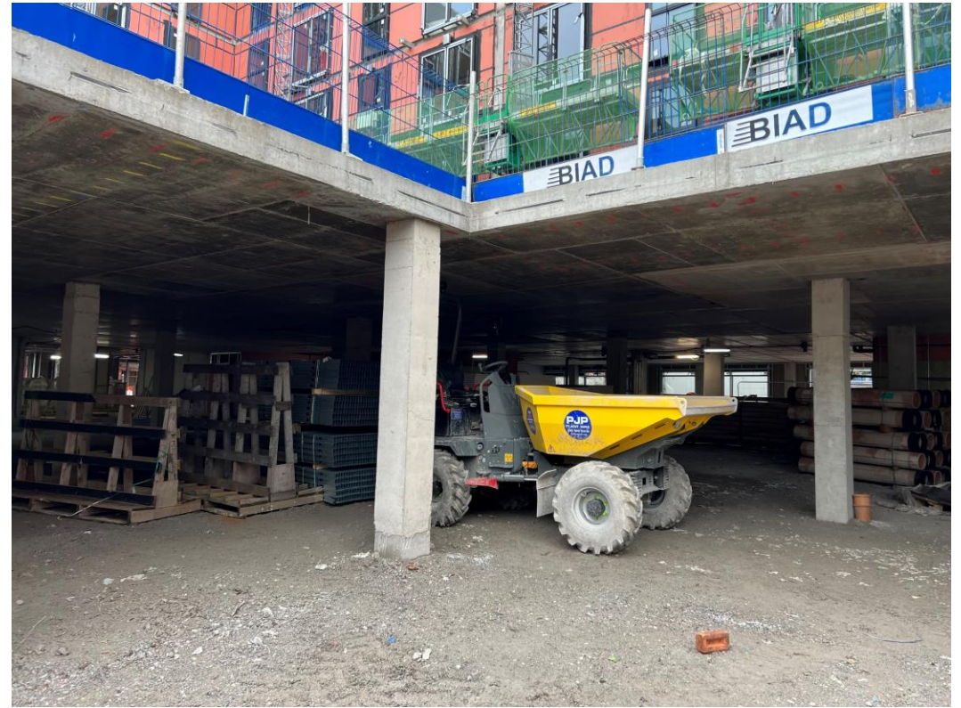
Block B – Podium complete
