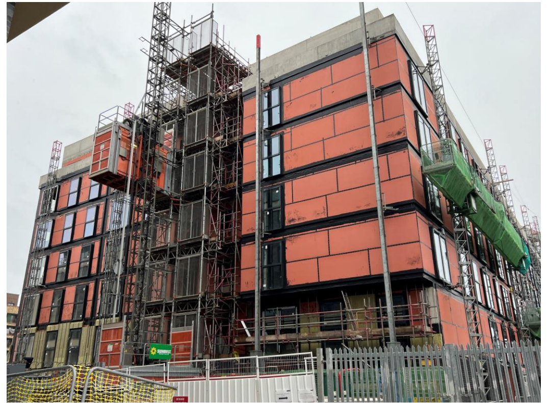
Ordsall Lane site view
