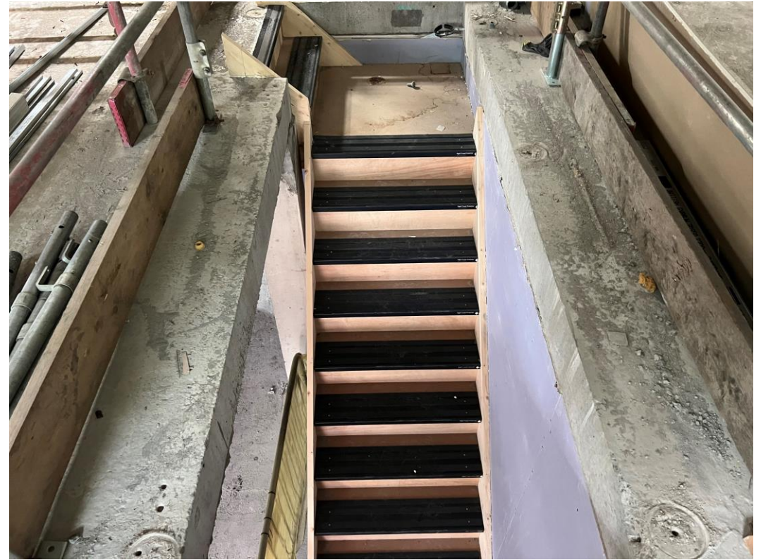
Upper levels timber staircase
