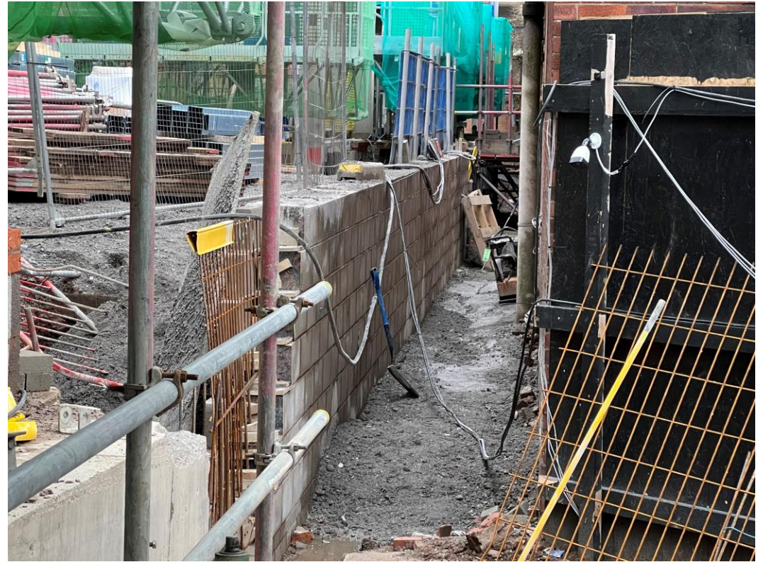
Block B – Retaining wall structure
