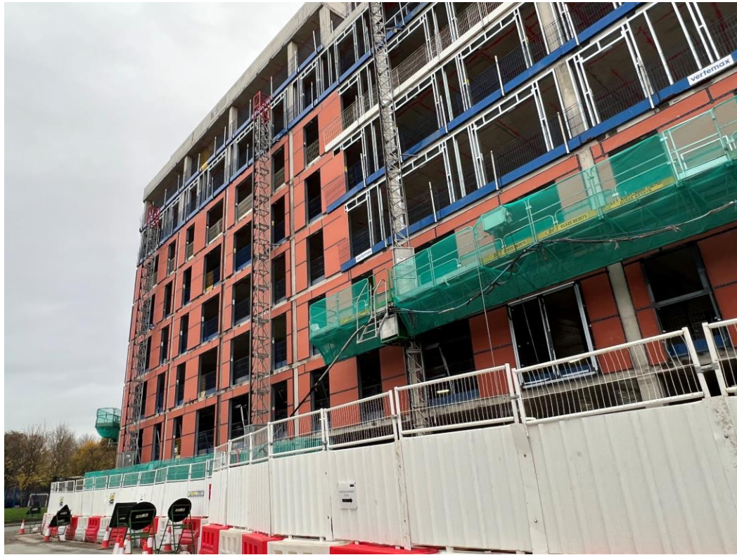
Ordsall Lane site view
