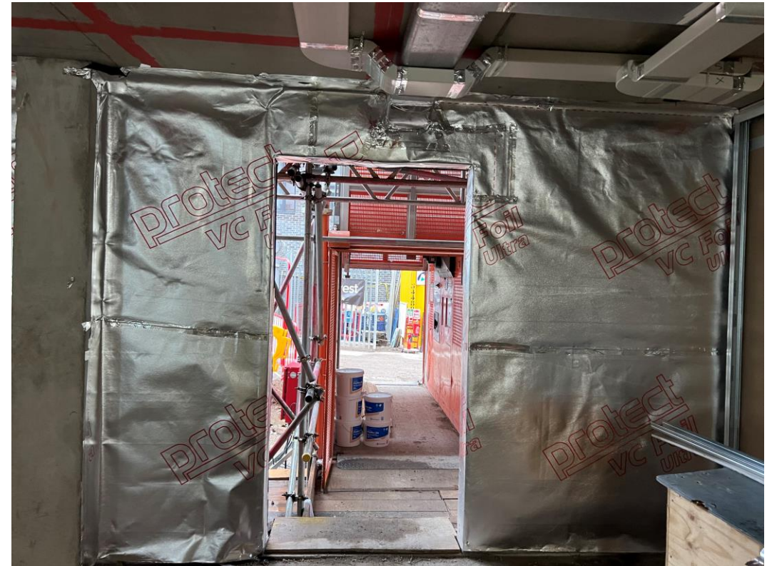
Ground floor partition & VCL external
