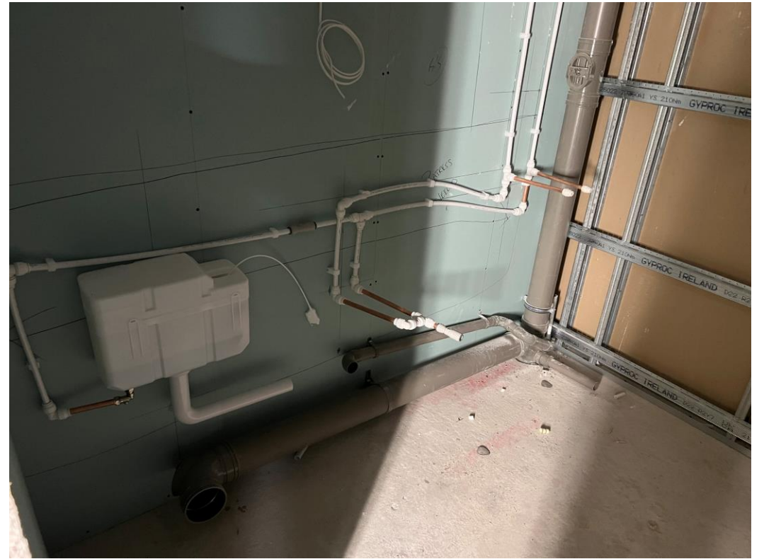
Upper level Apartment 1 st fix sanitary
