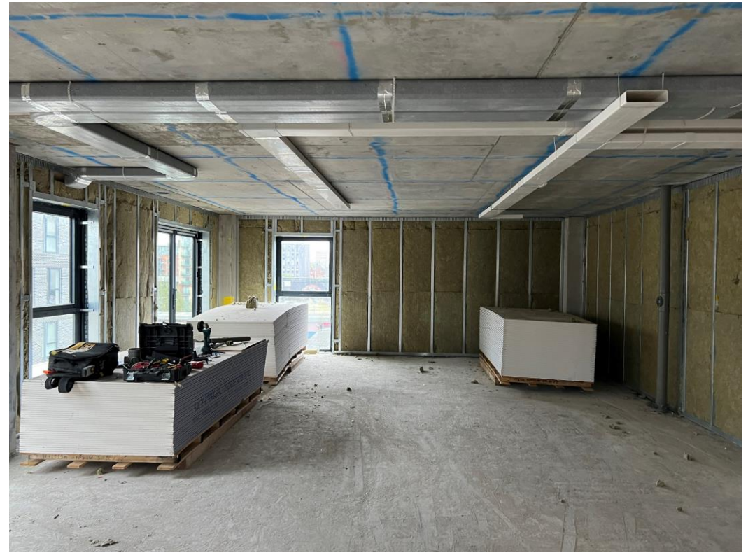
Upper levels drainage and mechanical ducting, windows installed
