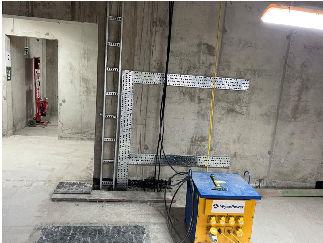
Upper level electrical works commenced
