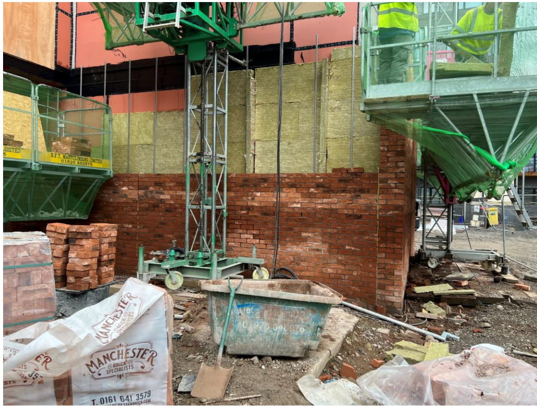
Block B – External brickwork construction
