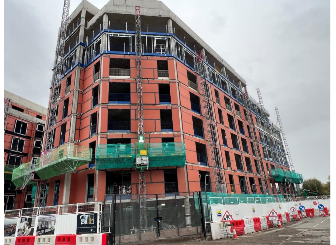
Ordsall Lane site view
