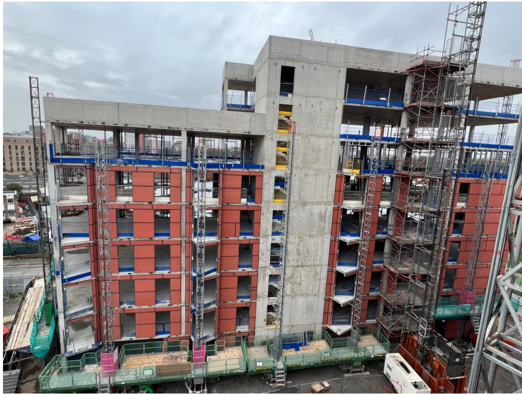
Block A – SFS & weatherboarding installed
