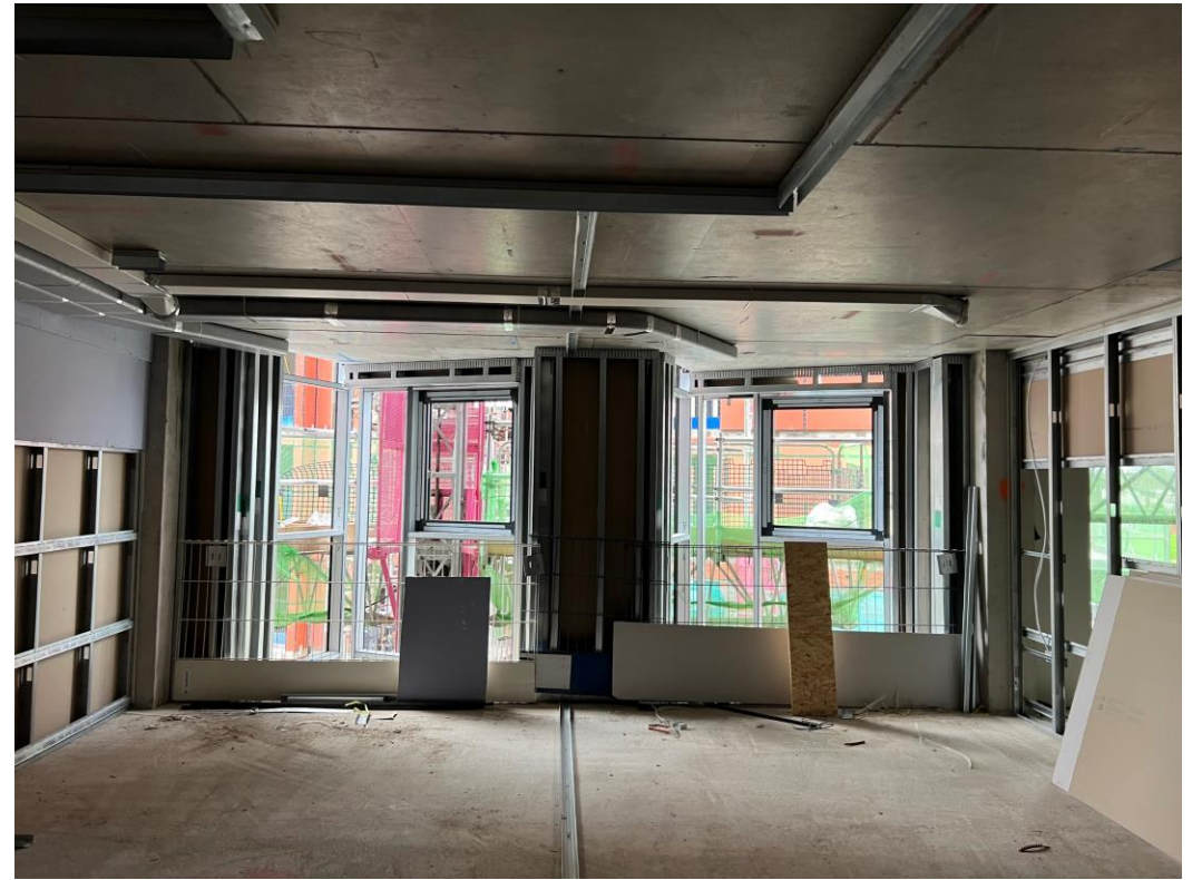
Upper levels partition wall framework
