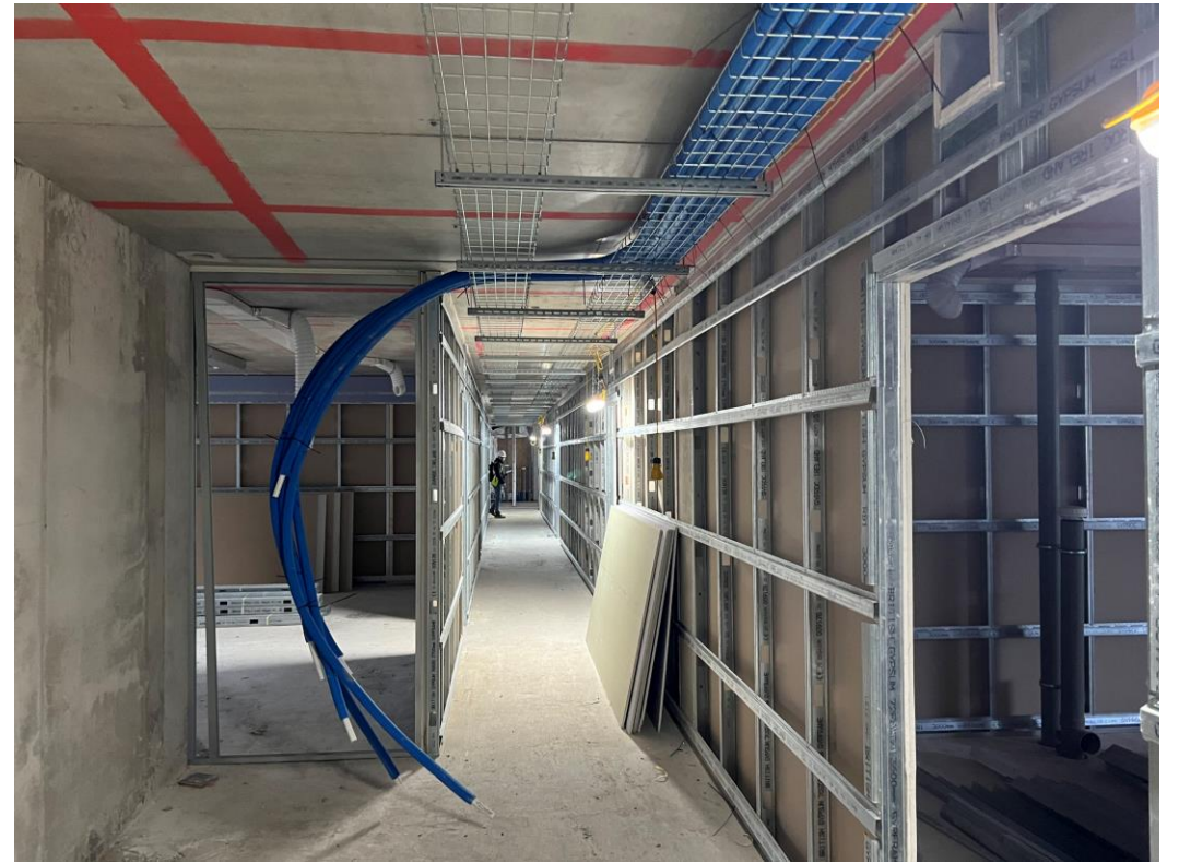
Upper level Corridor partition walls & services
