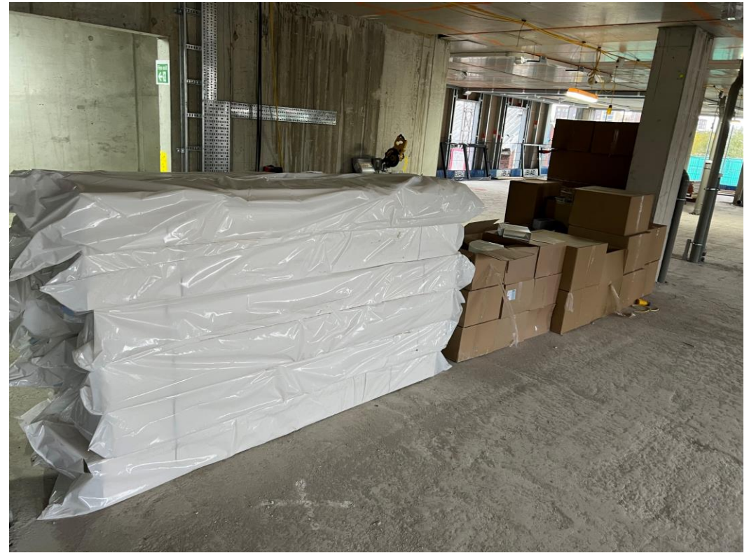
First floor mechanical plant materials stored
