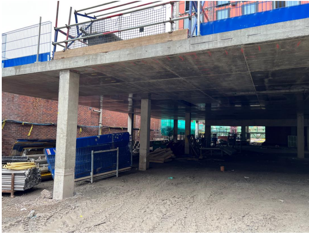
Block B – Podium complete
