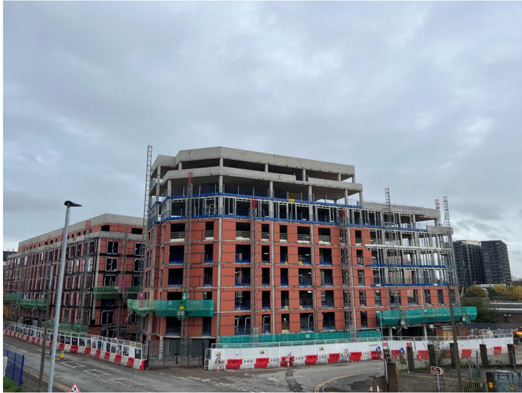
Ordsall Lane site view
