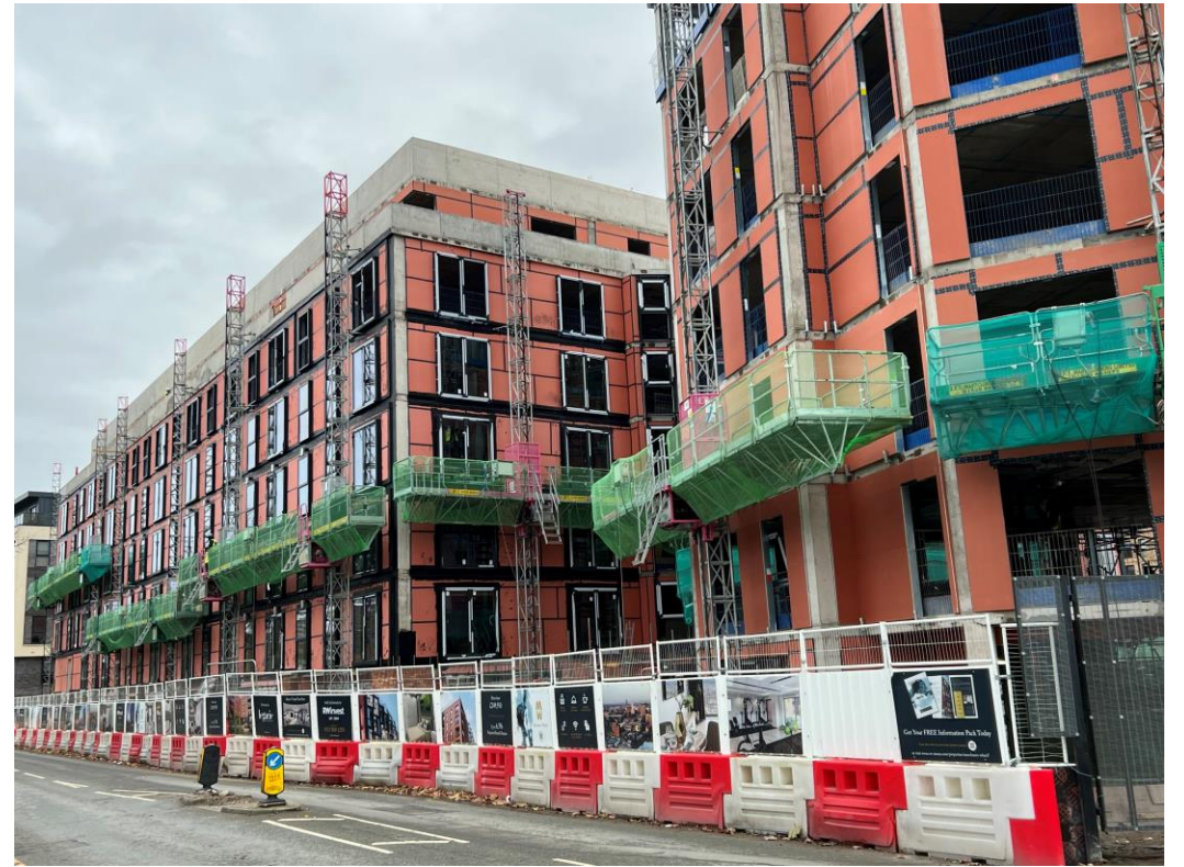
Ordsall Lane site view
