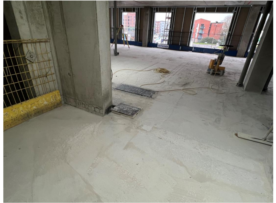
Upper level floor slab preparation
