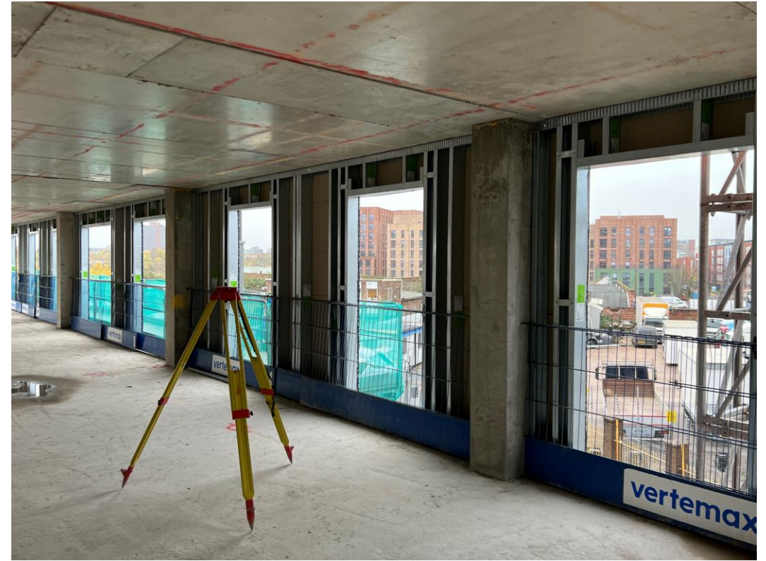
Upper level Setting out partitions due to commence
