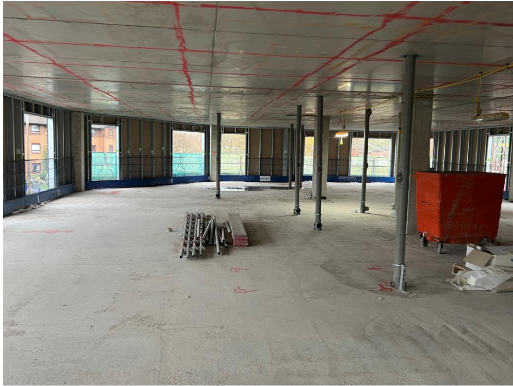
Upper level SFS and weatherboarding
