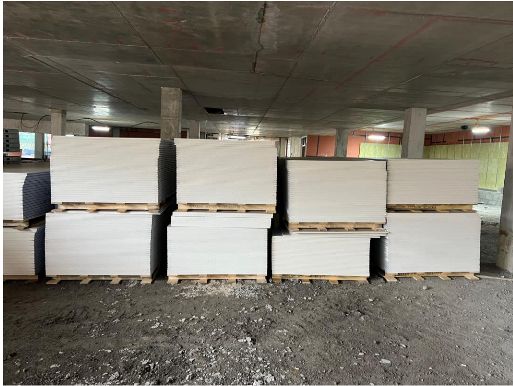
Ground floor undercroft
