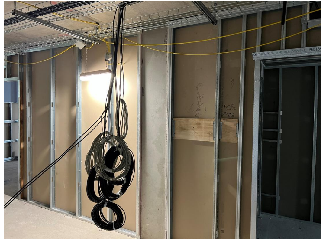
Upper level Corridor partition walls & services
