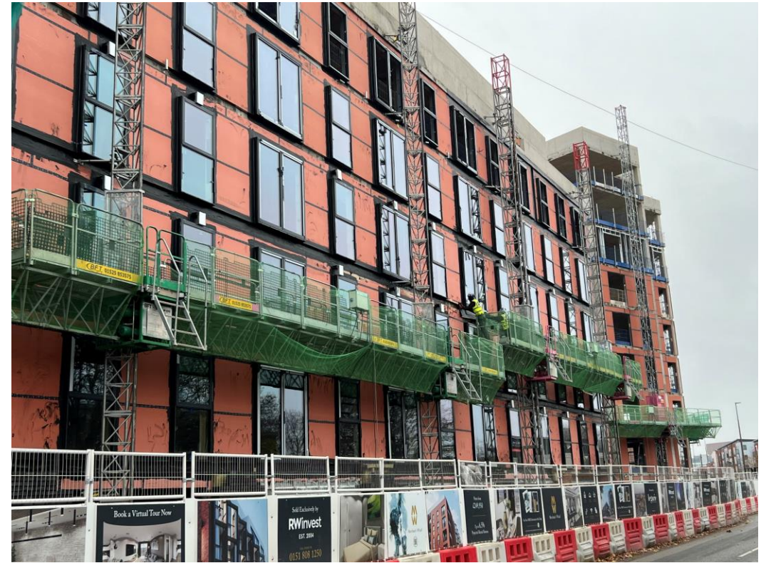
Ordsall Lane site view
