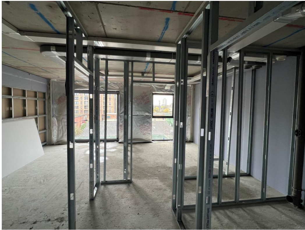
Upper levels partition wall framework
