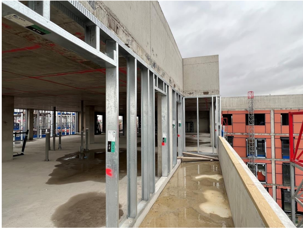
Block B – Roof balcony & parapet structure
