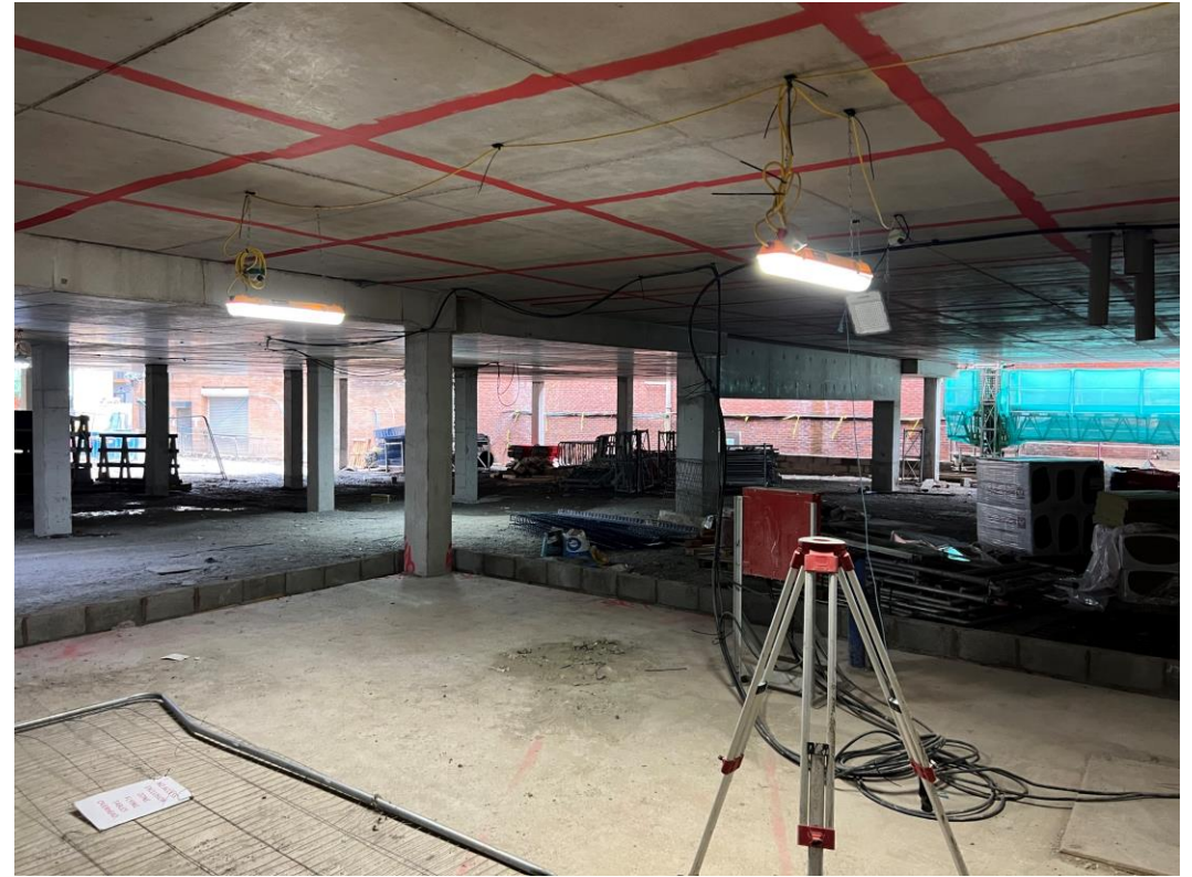
Ground floor undercroft
