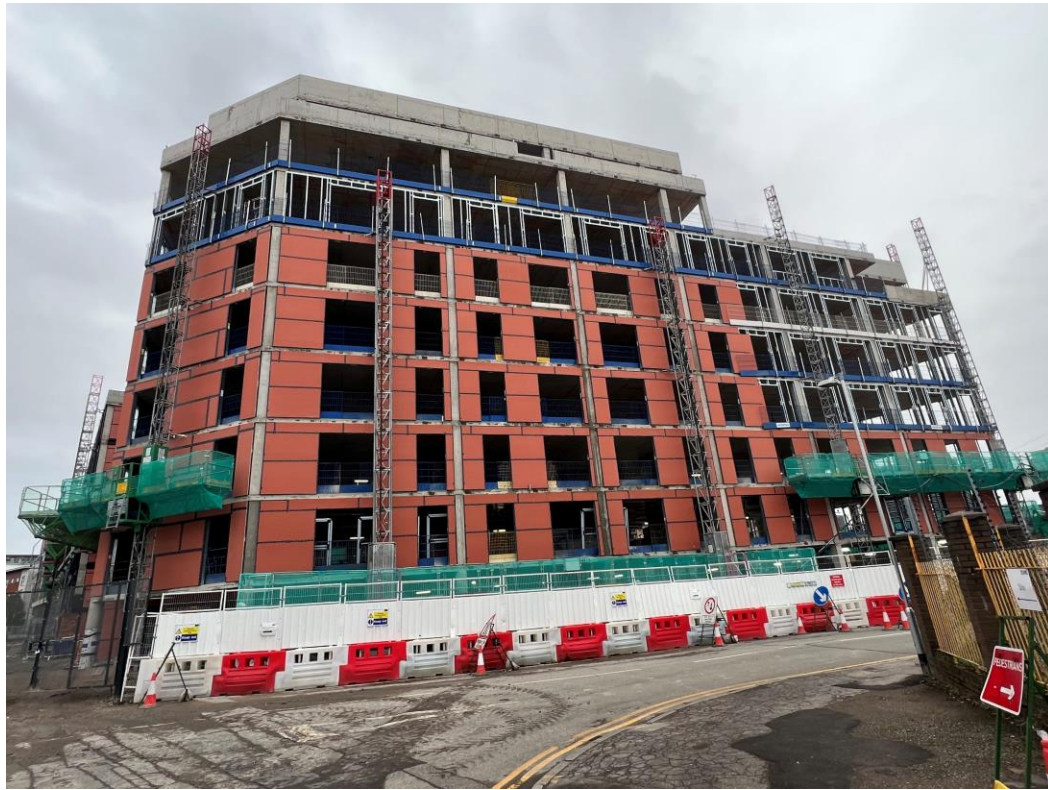
Ordsall Lane site view
