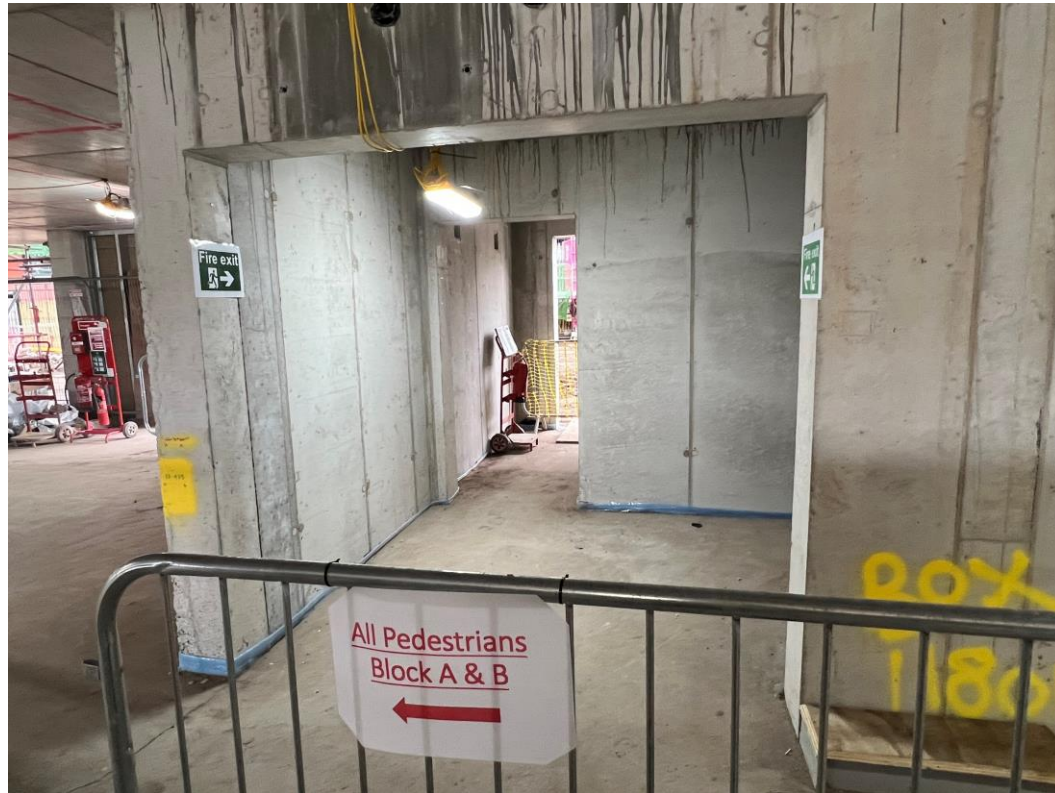
Ground floor lift core and stairwell
