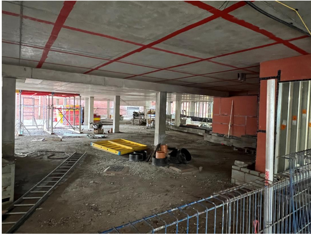
Ground floor undercroft
