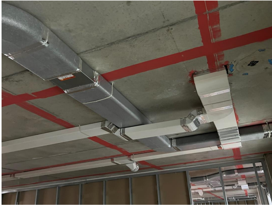
Ground floor drainage & 1 st fix mechanical
