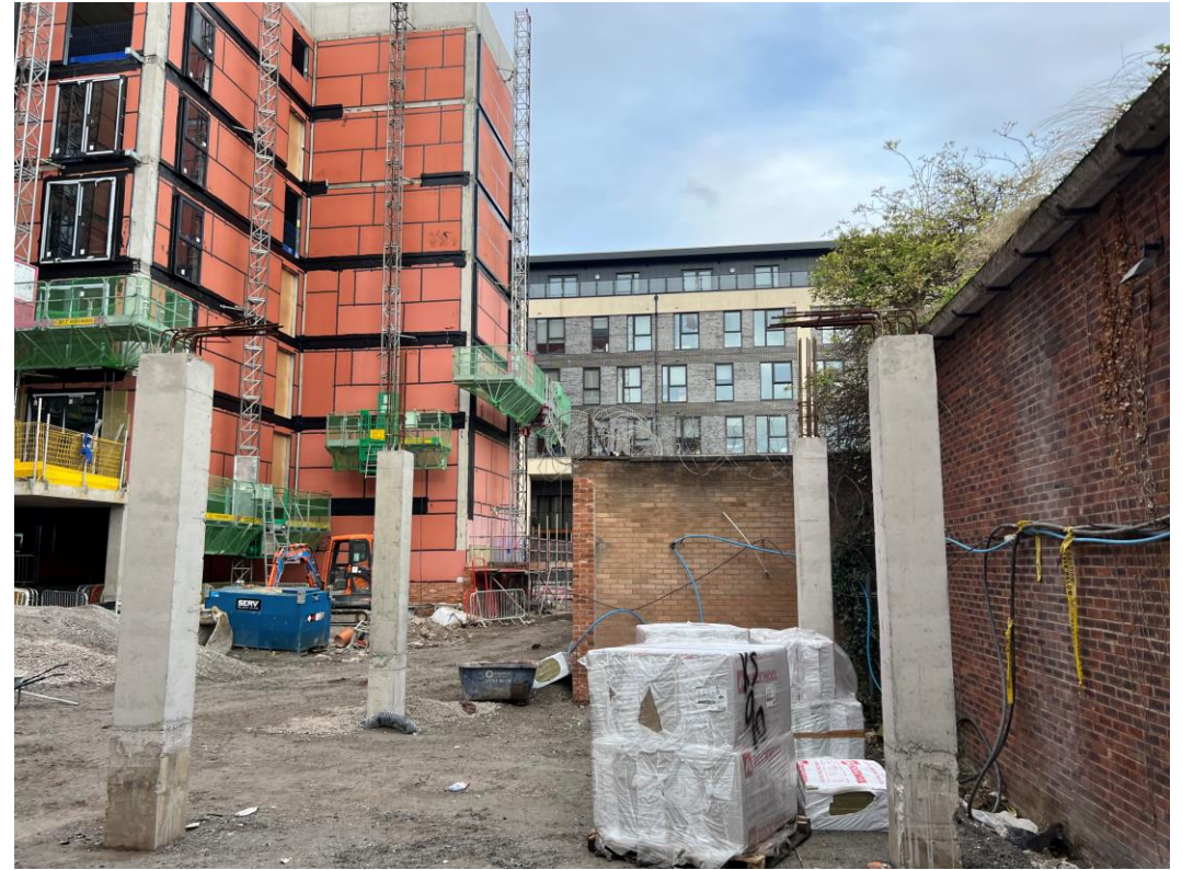
Block B – Podium construction
