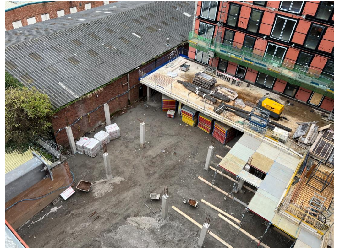
Block B – Podium construction
