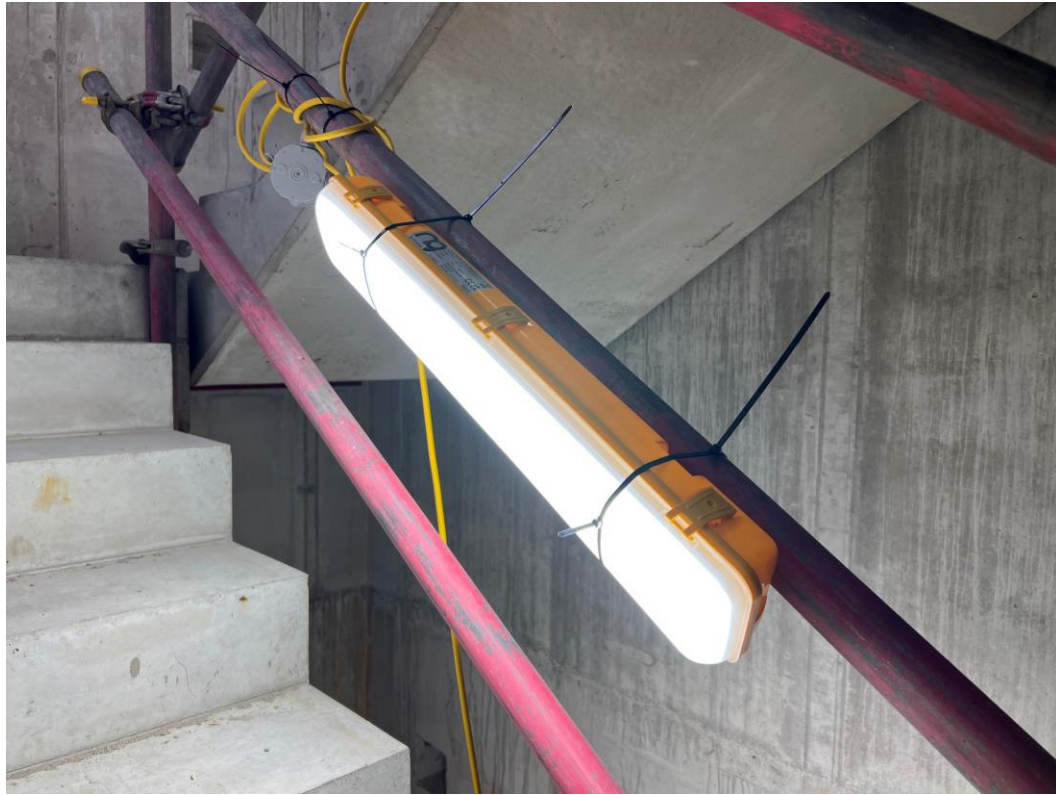
Temporary lighting installed
