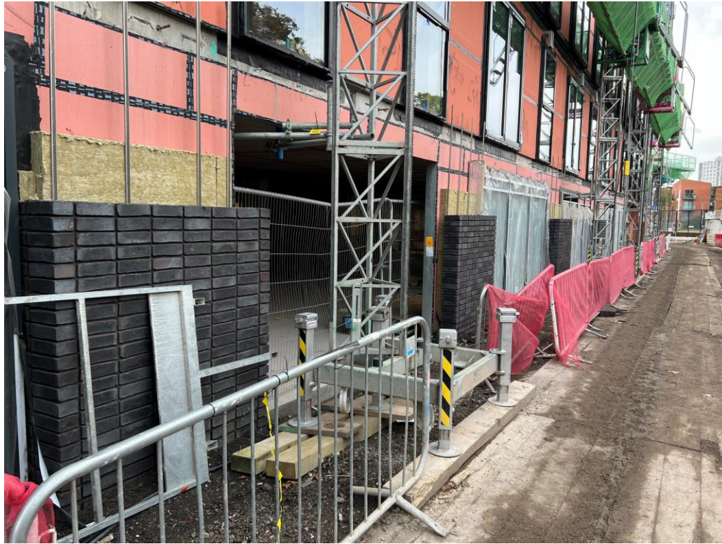
Block B – External brickwork construction
