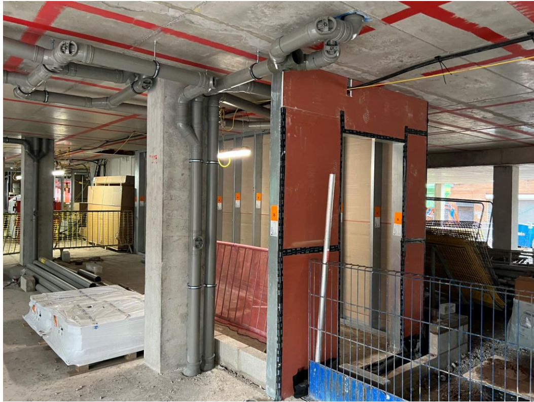
Ground floor partition walls
