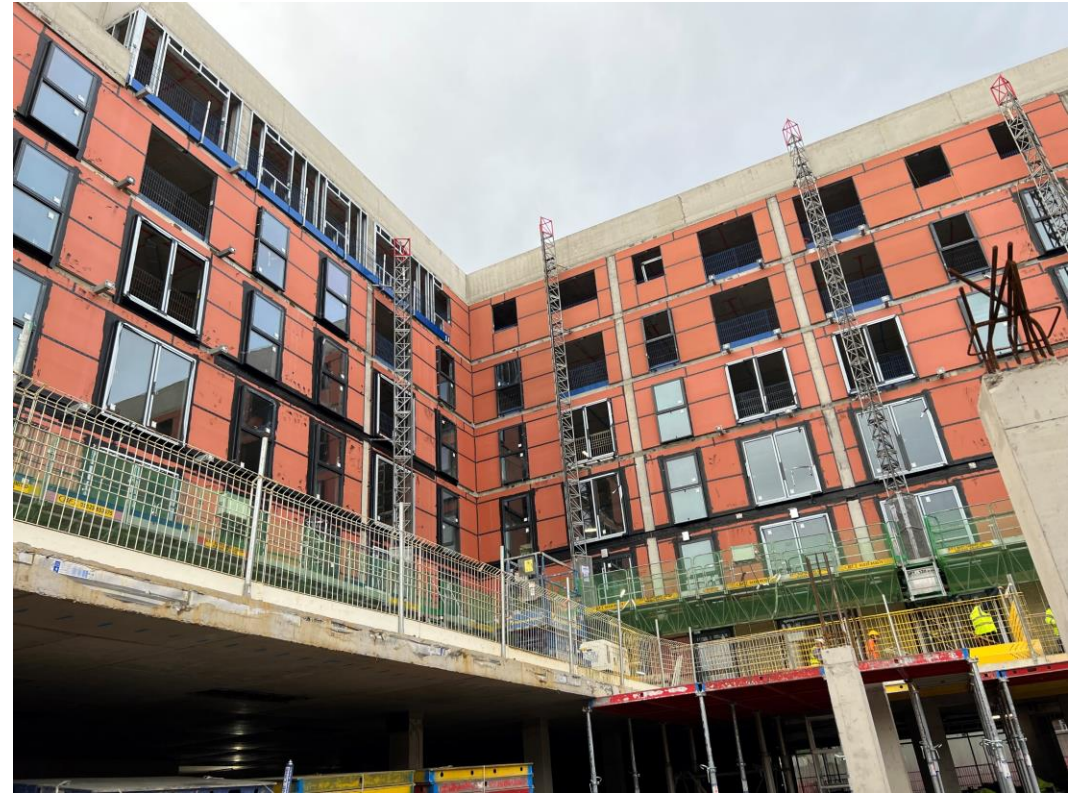
Block B – Podium construction
