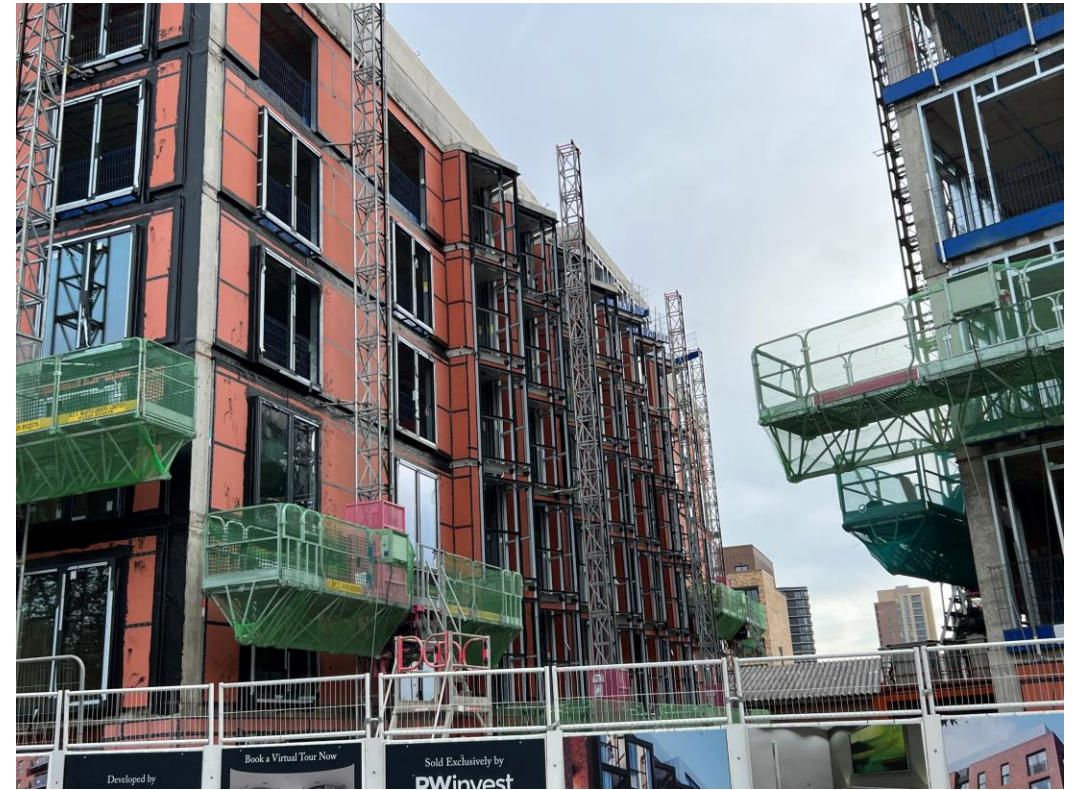
Ordsall Lane site view
