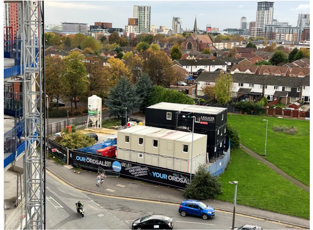
Site Accommodation Relocated Ordsall Lane /Worrall Street
