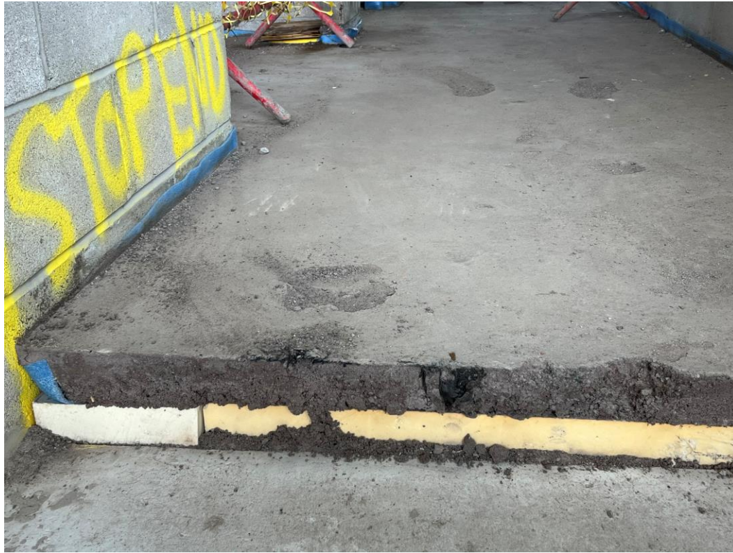
Ground floor insulation and screed
