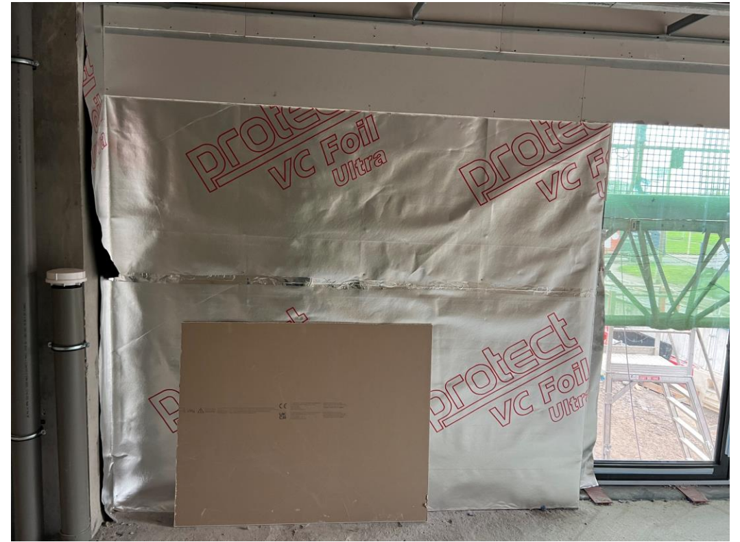
First floor Apartment external wall VC layer
