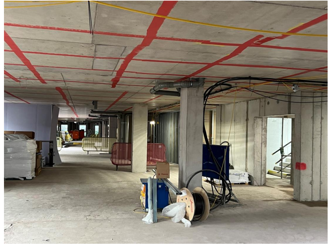
Ground floor drainage & 1 st fix mechanical
