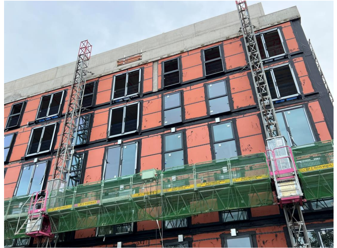
Ordsall Lane site view
