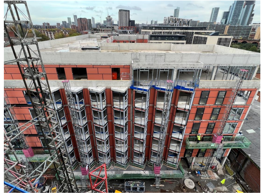
Block B – Weatherboarding, windows & doors installed
