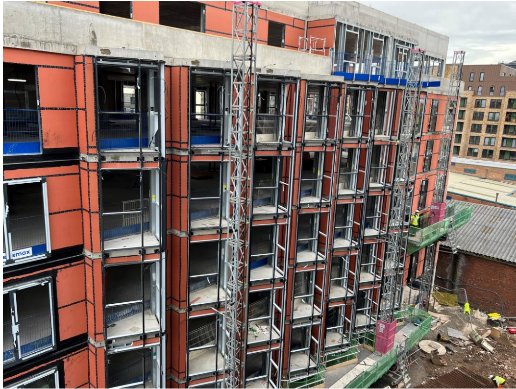
Block B – Weatherboarding, windows & doors installed
