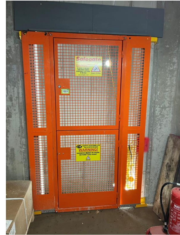
Ground floor lift shaft security gate
