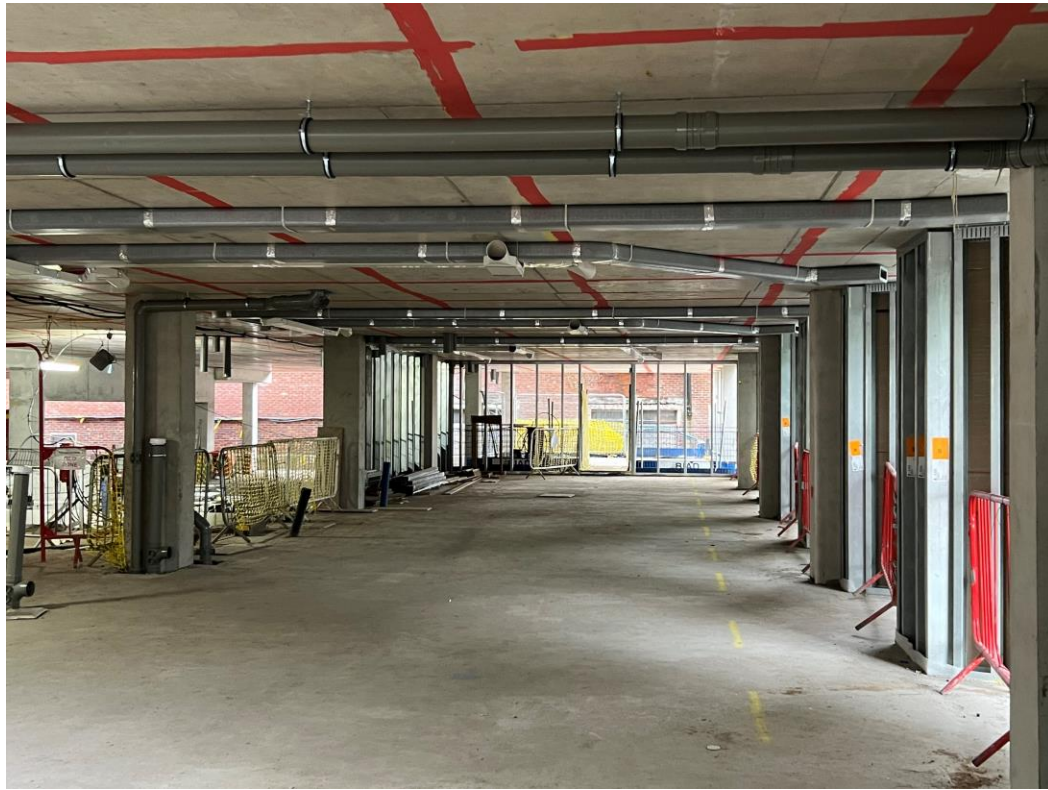
Ground floor drainage & 1 st fix mechanical
