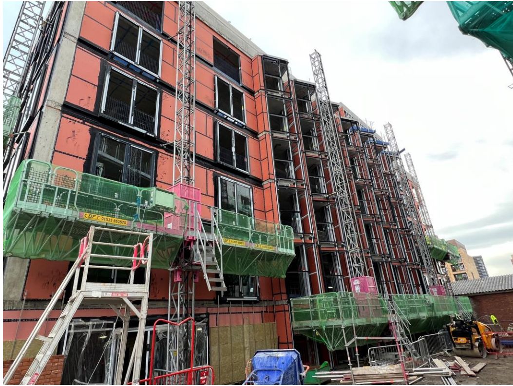
Block B – Weatherboarding, windows & doors installed
