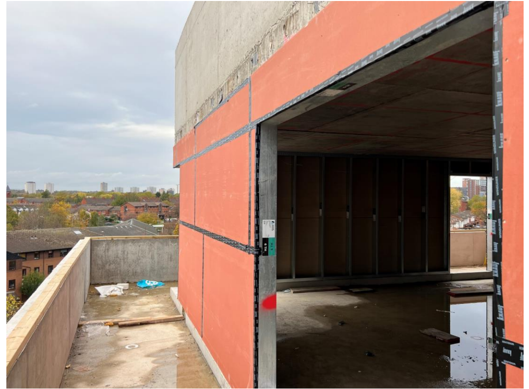
Block B – Balcony & parapet structure
