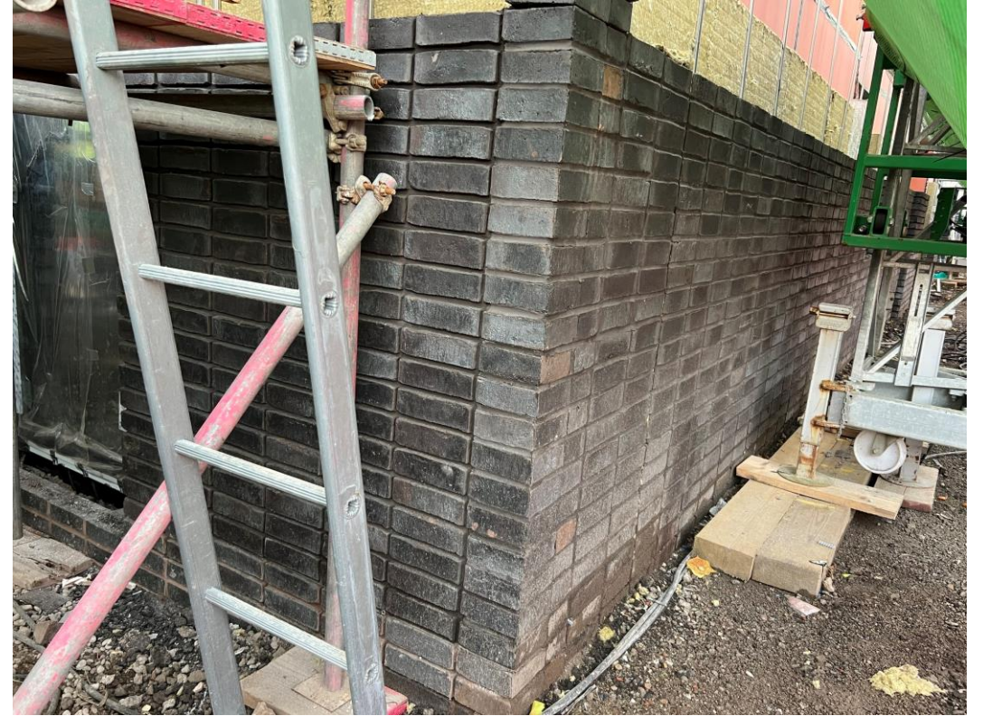
Block B – External brickwork construction
