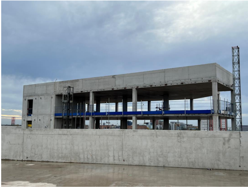
Block A – Roof & parapet structure
