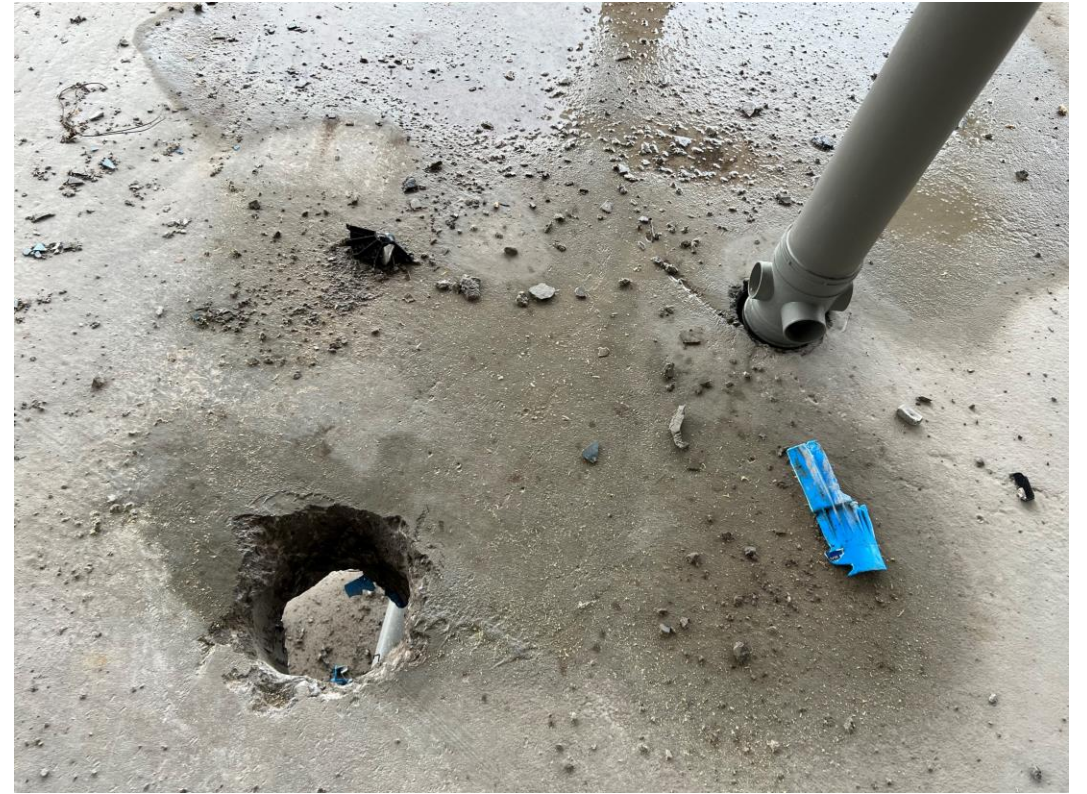
Upper floor core drilling drainage
