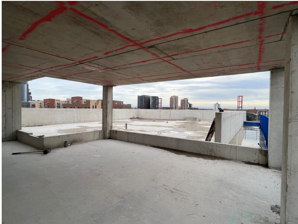
Upper floor concrete framework
