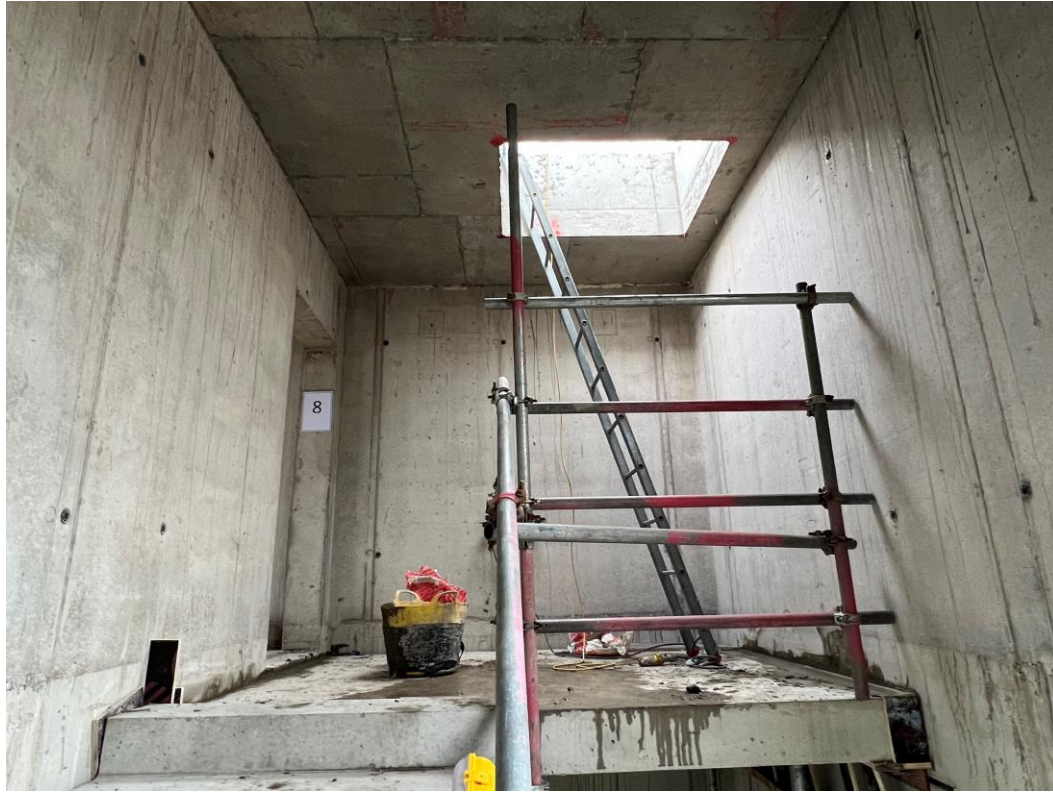
Upper floor landing
