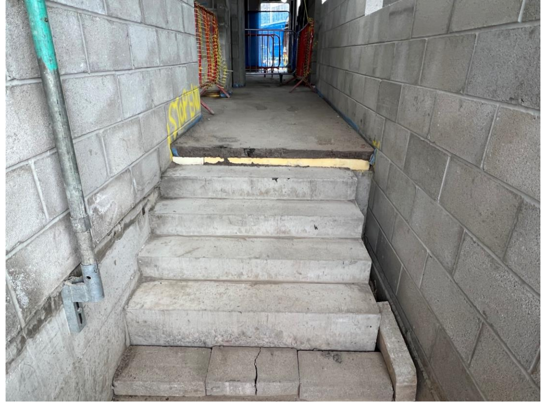
Concrete steps rear entrance
