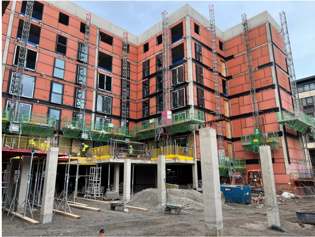
Block B – Podium construction
