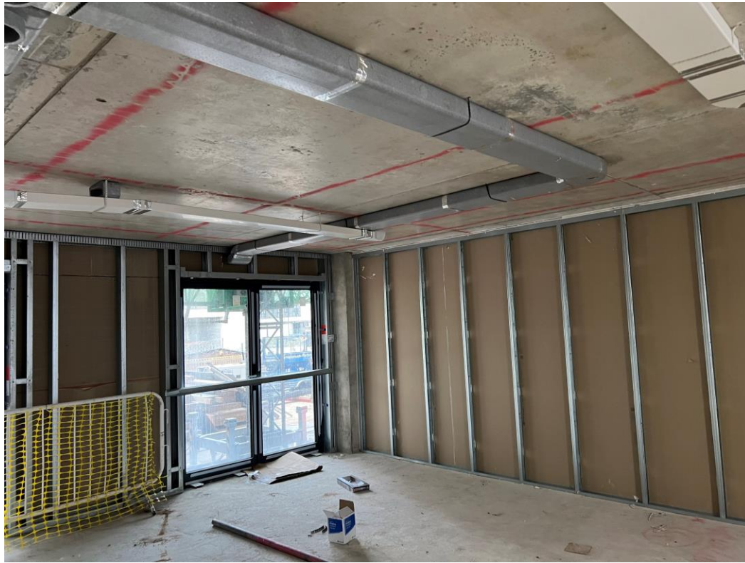
First floor Apartment 1 st fix mechanical & partition walls formed
