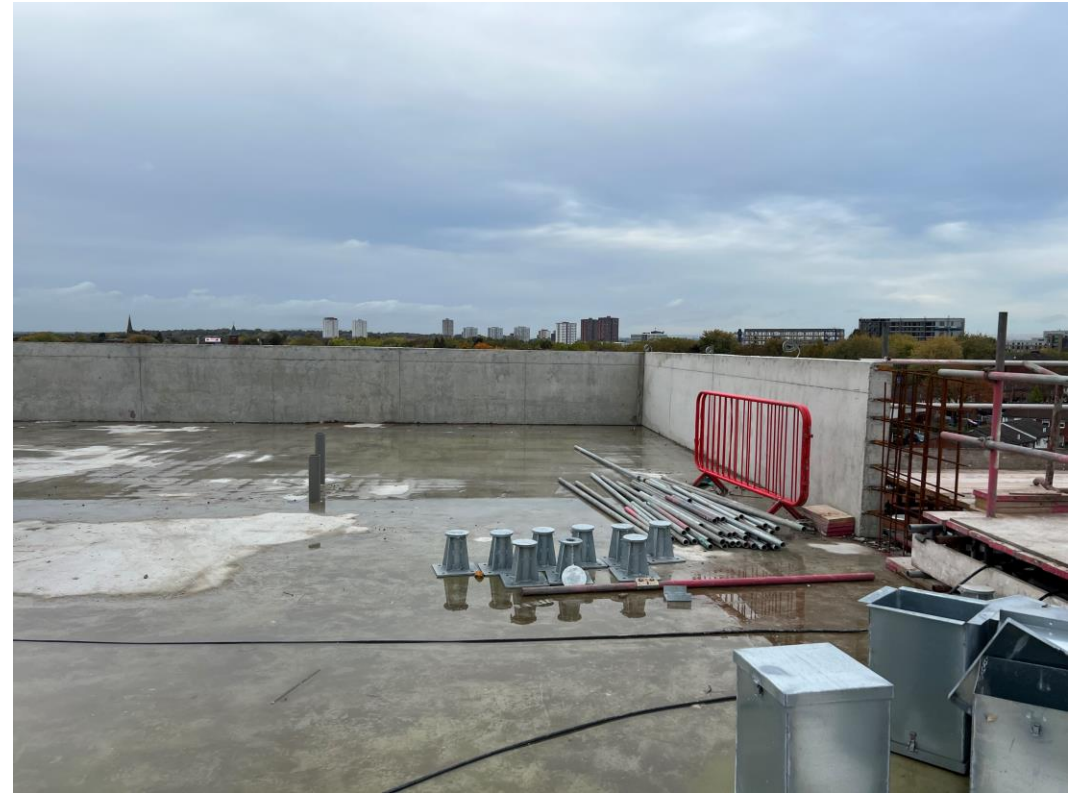
Block B – Roof & parapet structure
