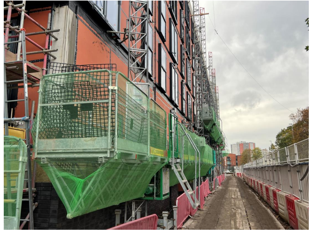
Block B – Weatherboarding, windows & doors installed
