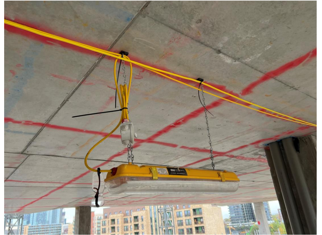
Temporary lighting installed
