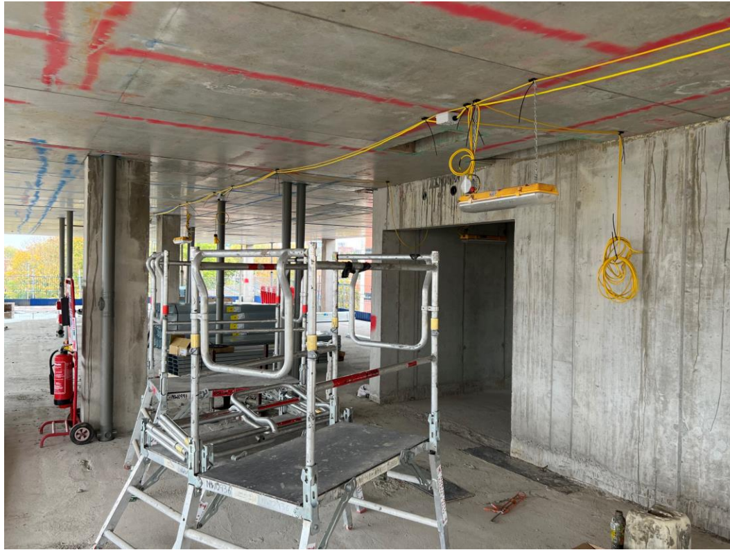
Temporary lighting installed
