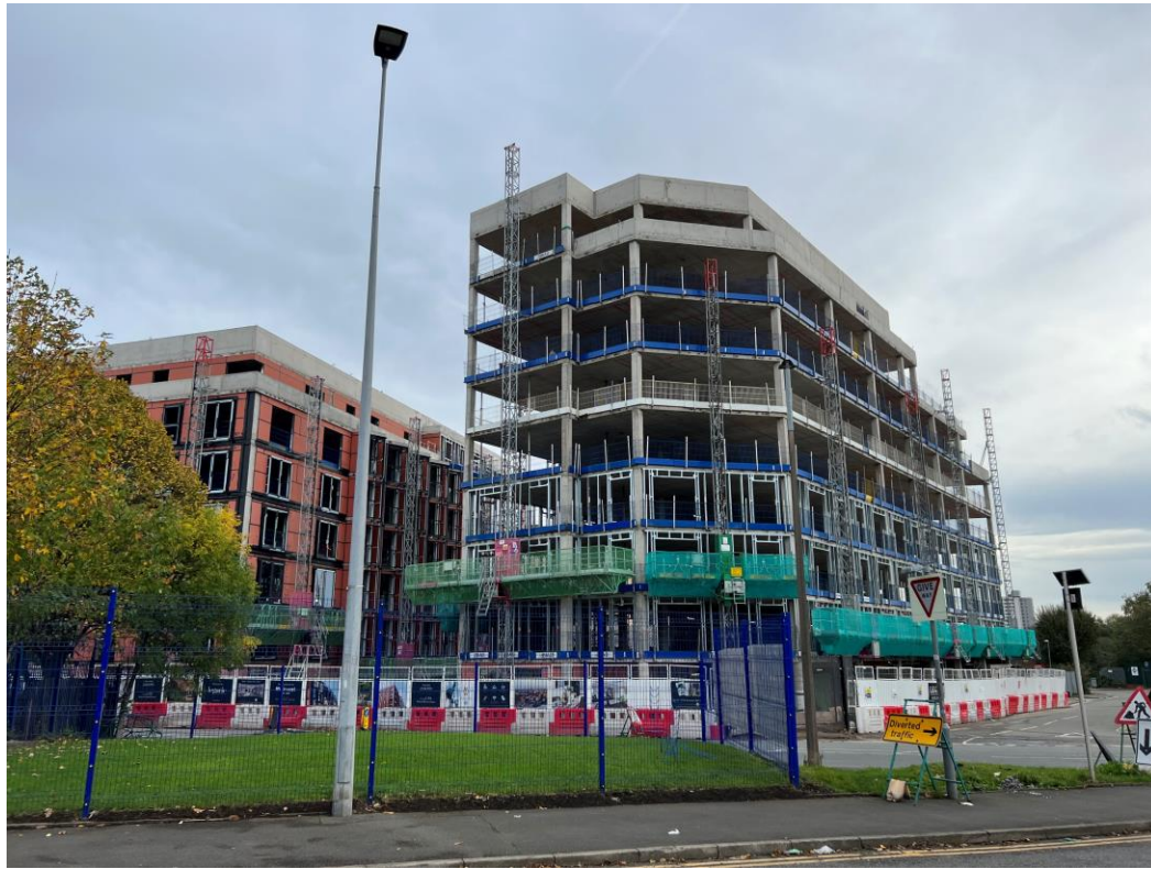
Ordsall Lane site view
