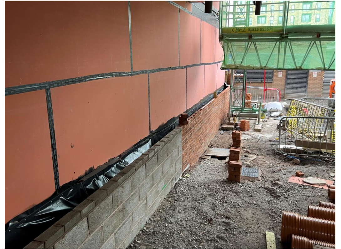
Ground floor undercroft
