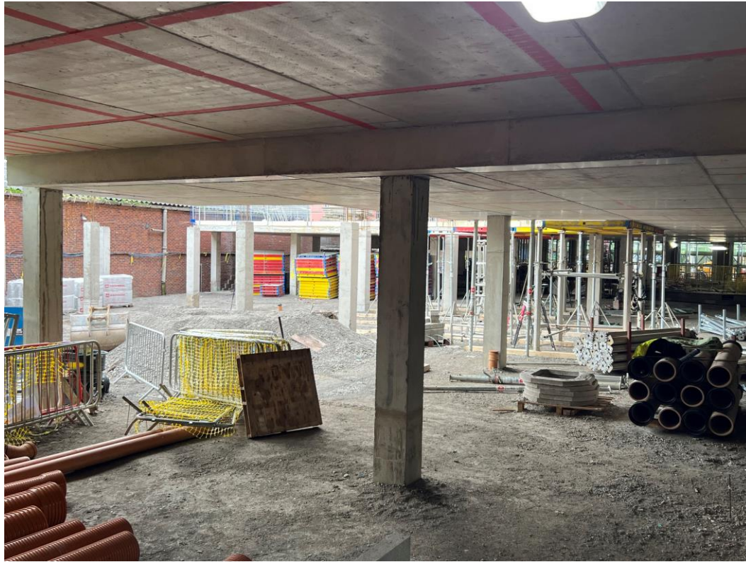
Block B – Undercroft Podium construction
