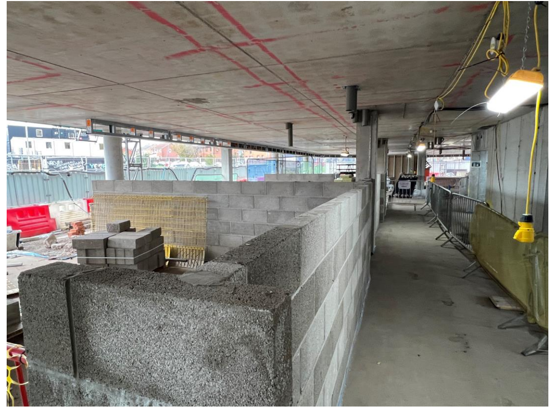
Ground floor blockwork
