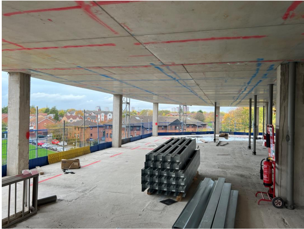
Upper floor concrete framework
