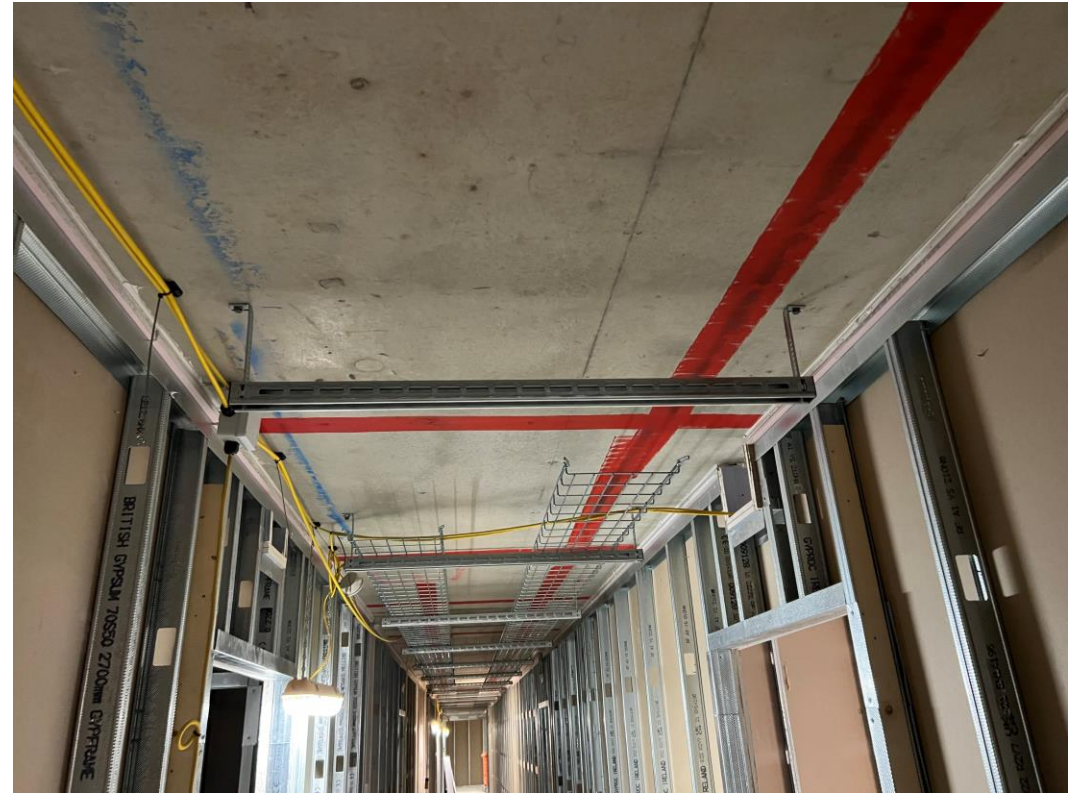
Second floor 1 st fix electrical & partition walls formed
