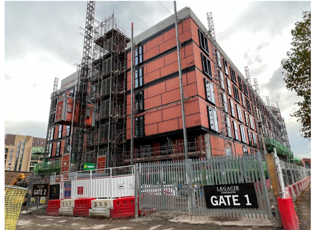
Ordsall Lane site view
