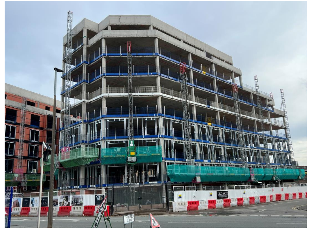
Ordsall Lane site view
