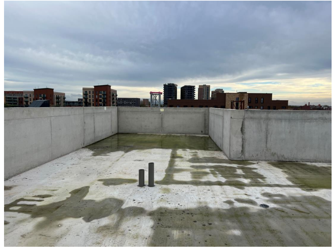
Block B – Roof & parapet structure
