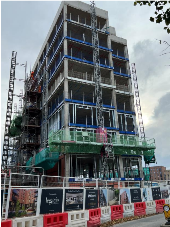
Ordsall Lane site view
