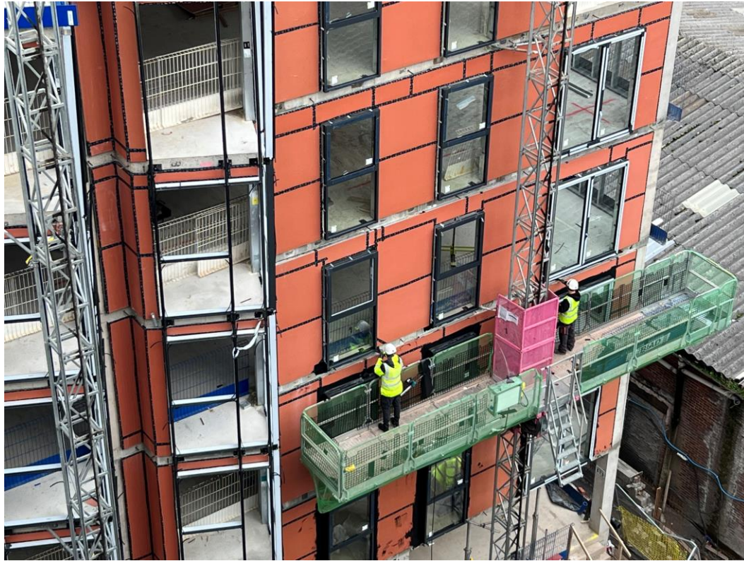
Block B – Weatherboarding, windows & doors installed
