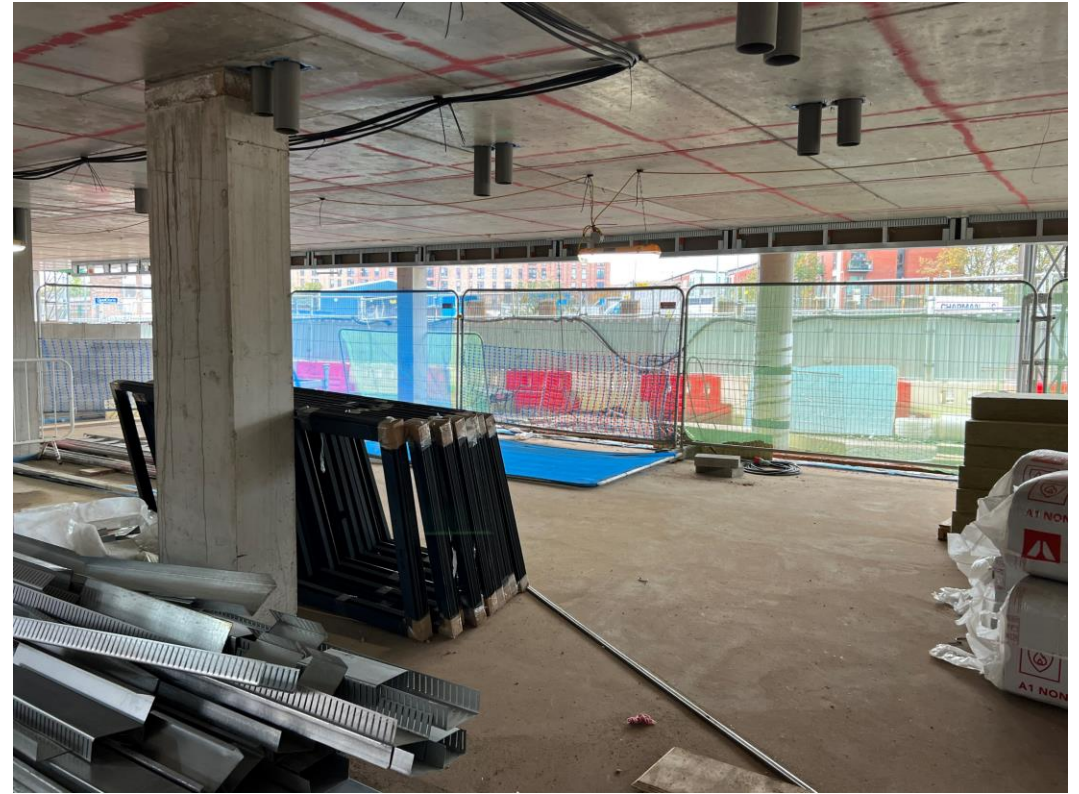
Ground floor insulation and screed
