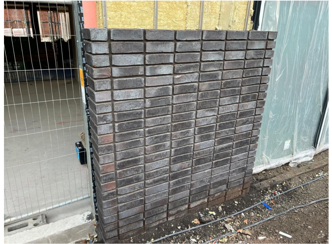
Block B – External brickwork construction
