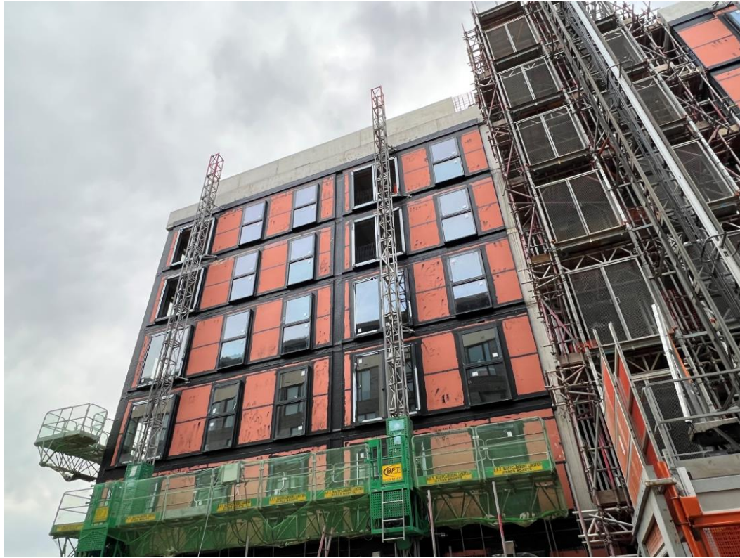
Block B – Weatherboarding, windows & doors installed
