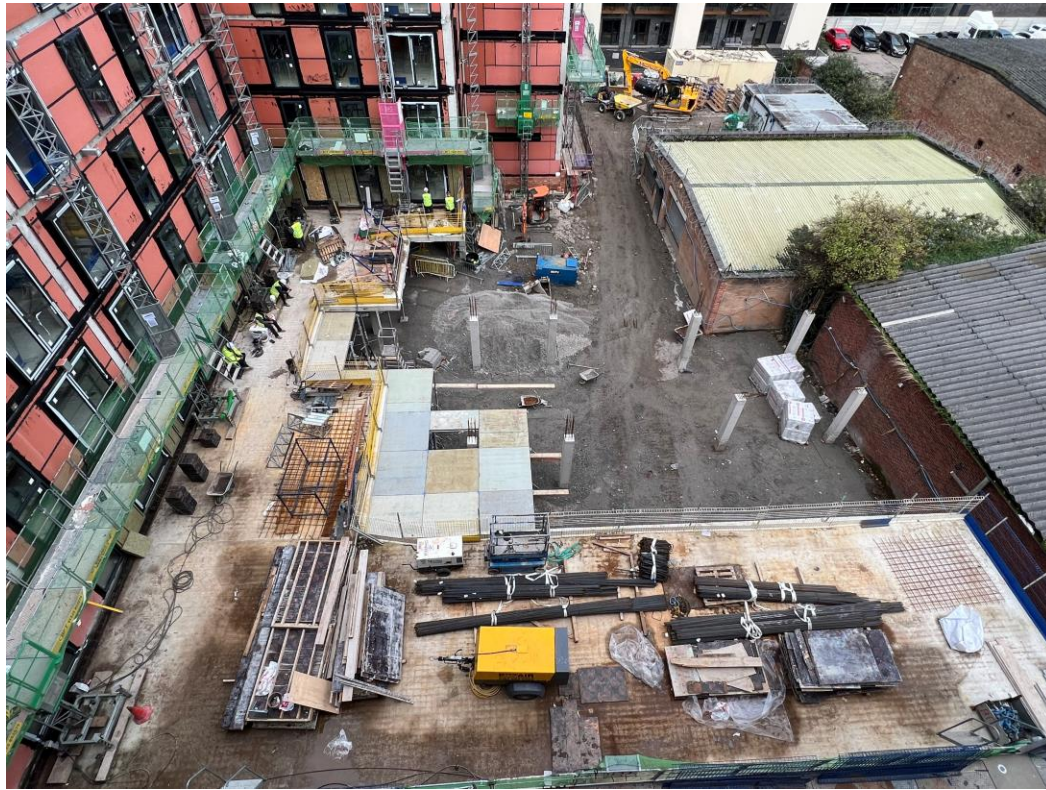
Block B – Podium construction
