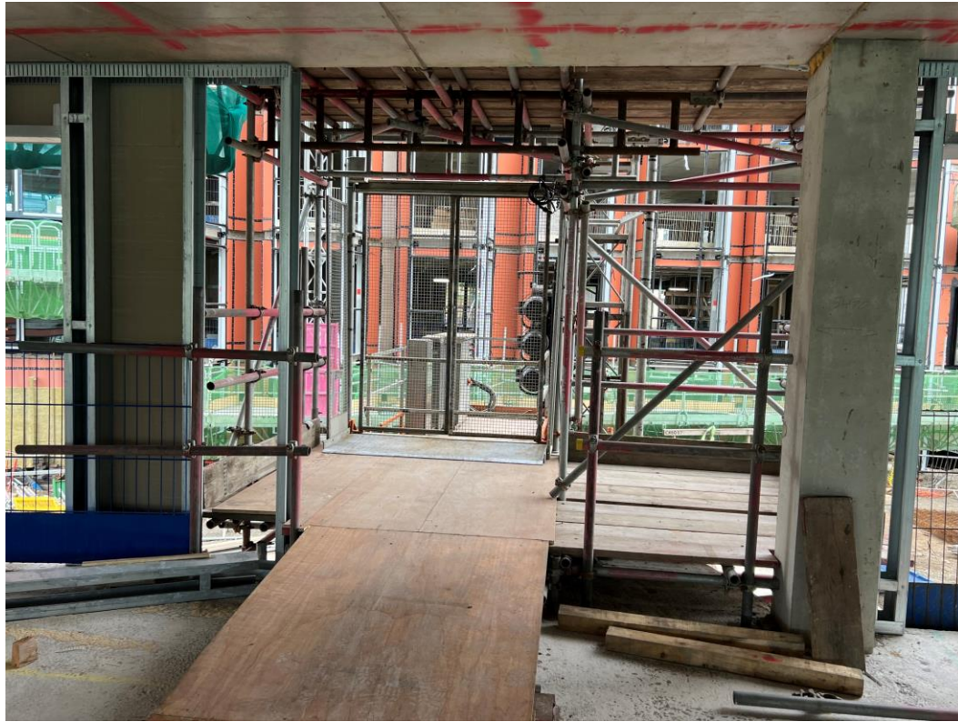
Upper floors hoist access
