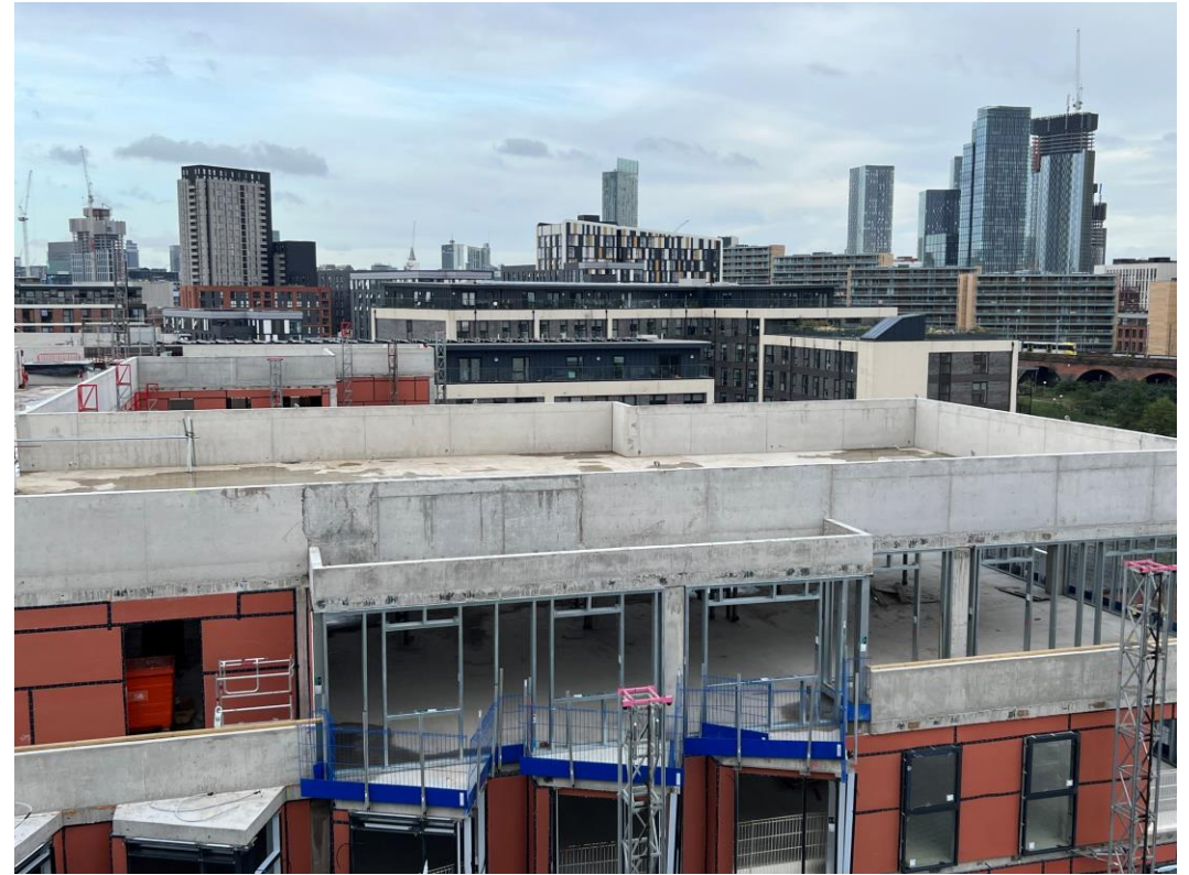
Block B – Weatherboarding, windows & doors installed
