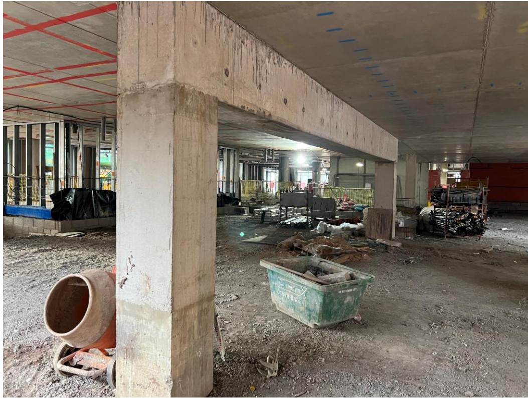
Ground floor undercroft
