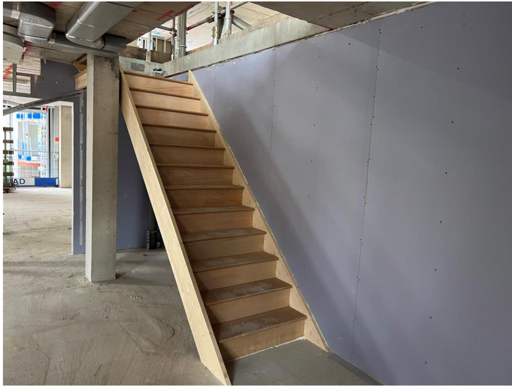
First floor timber staircase
