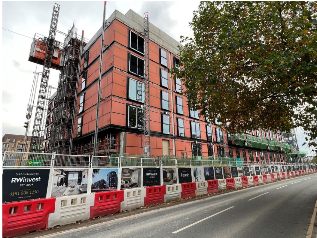
Ordsall Lane site view
