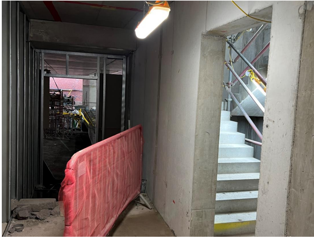
Ground floor partition walls
