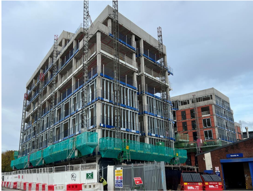
Worrall Street site view
