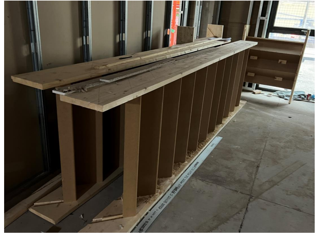
Ground floor timber staircase stored
