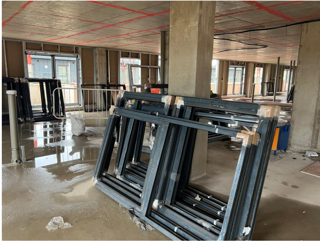
Upper floors Window frames stored
