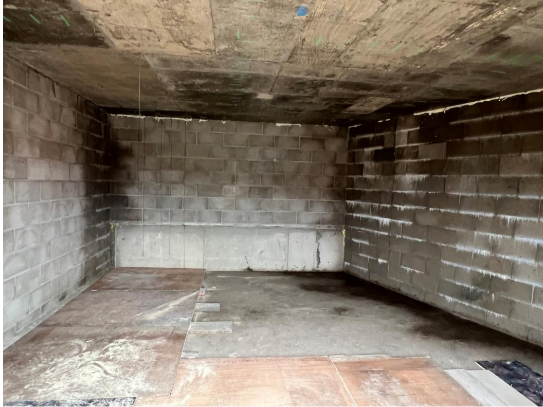
Ground floor plant room
