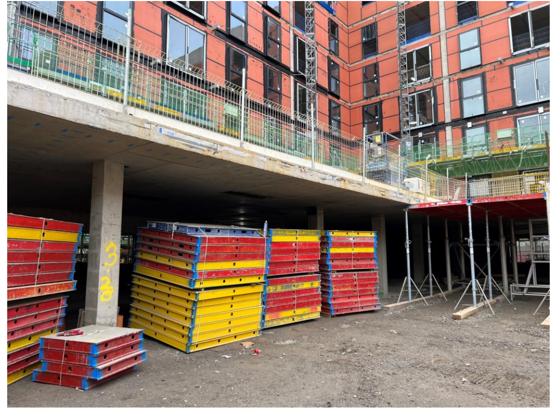
Block B – Podium construction
