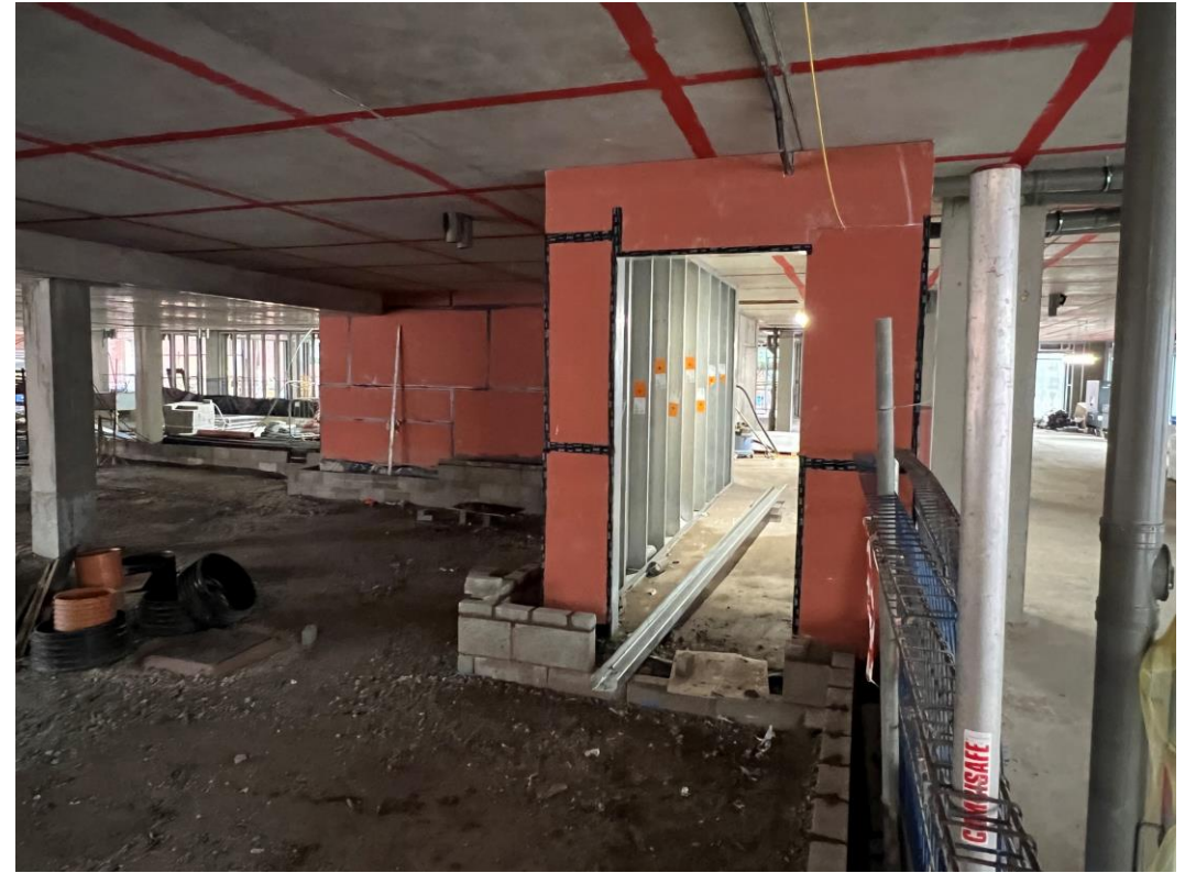
Ground floor partition walls
