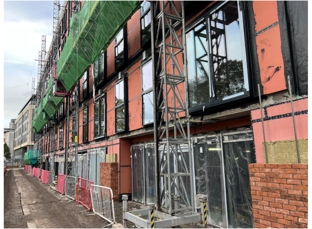
Block B – External brickwork construction
