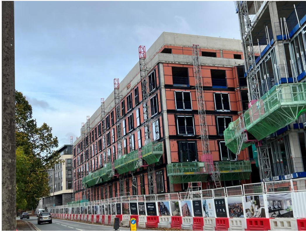
Ordsall Lane site view
