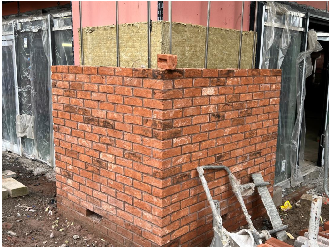
Block B – External brickwork construction
