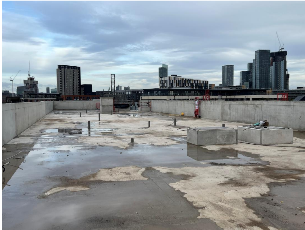
Block B – Roof & parapet structure
