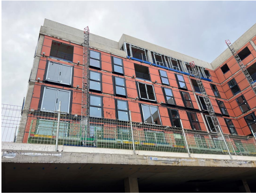
Block B – Podium construction
