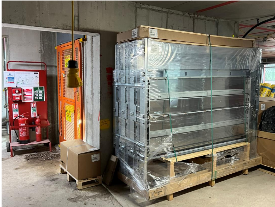
Ground floor smoke vent stored
