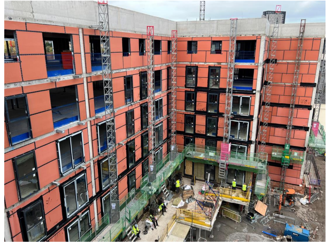
Block B – Weatherboarding, windows & doors installed
