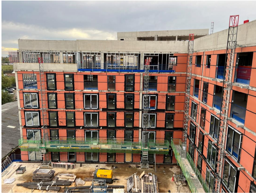
Block B – Weatherboarding, windows & doors installed
