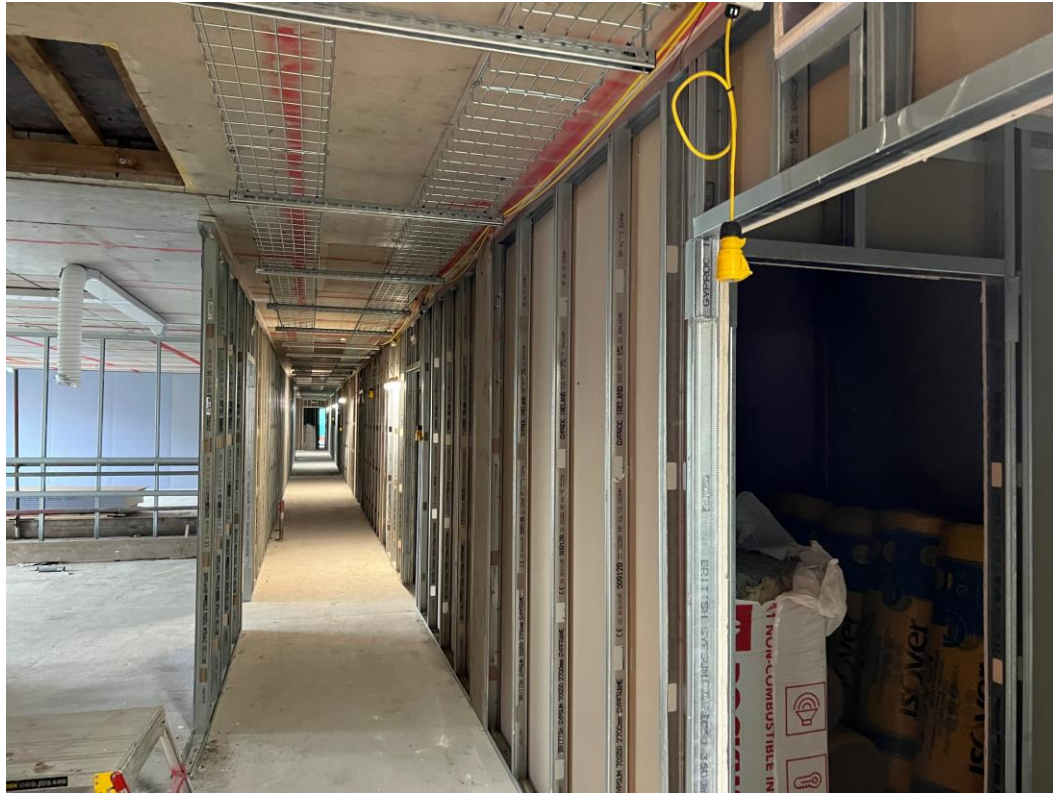
Second floor corridor 1 st fix electrical & partition walls formed
