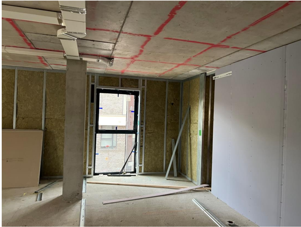
Second floor Apartment 1 st fix mechanical & partition walls formed
