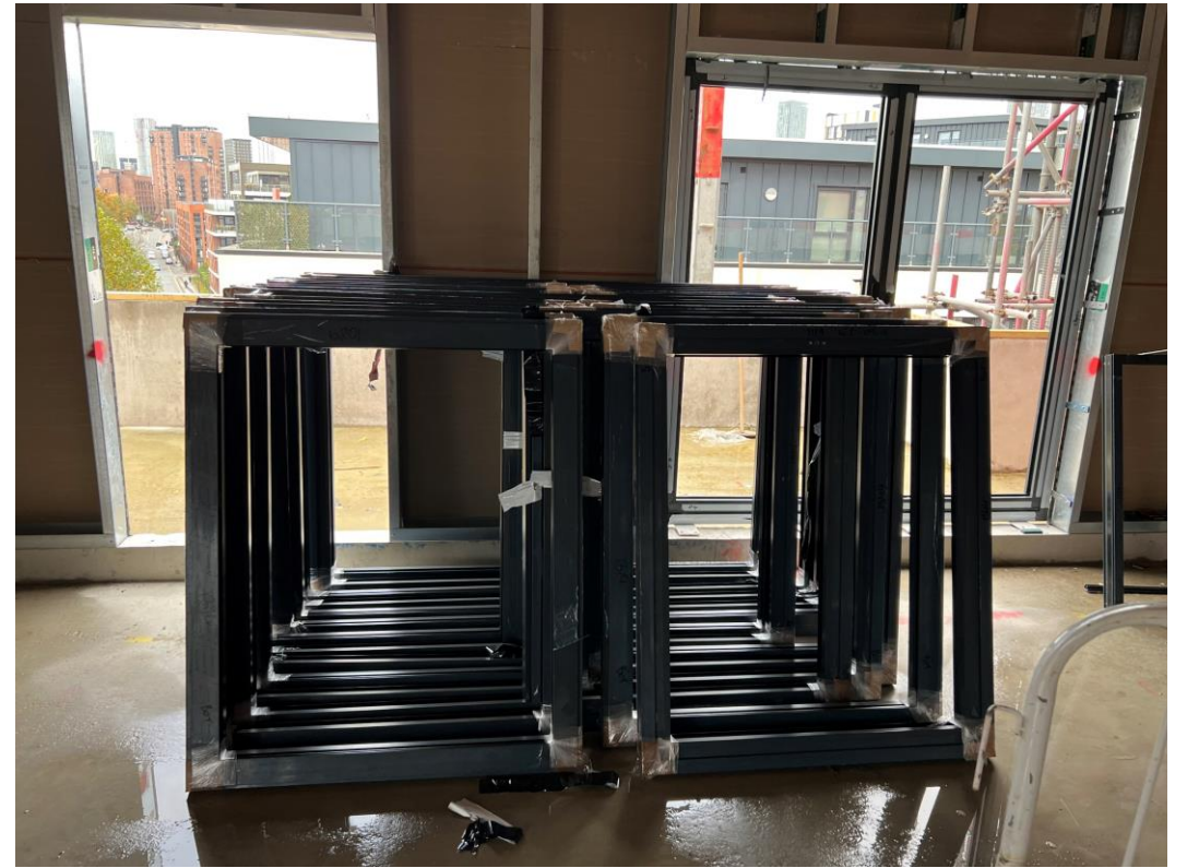
Upper floors Window frames stored
