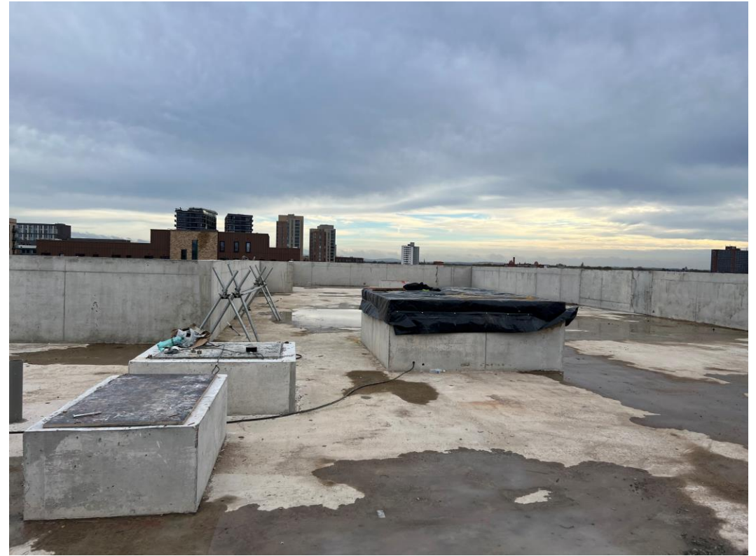
Block B – Roof & parapet structure
