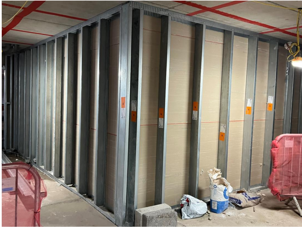
Ground floor partition walls
