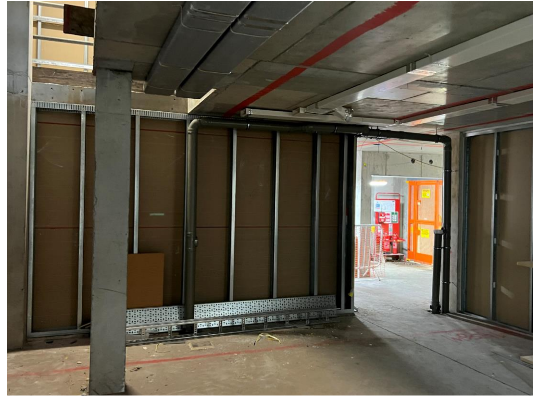
Ground floor partition walls
