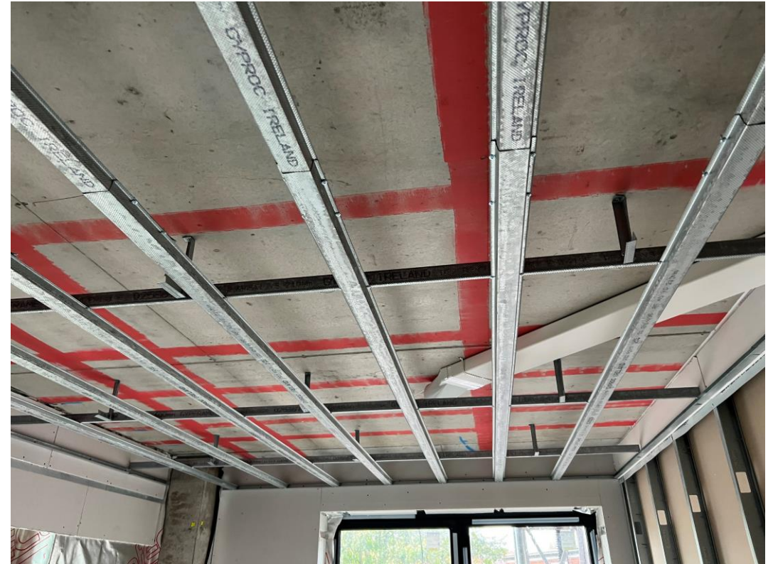
First floor Apartment suspended ceiling & partition walls formed
