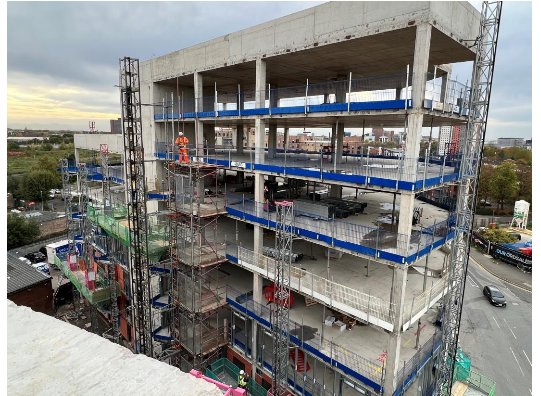
Block A – Concrete frame structure
