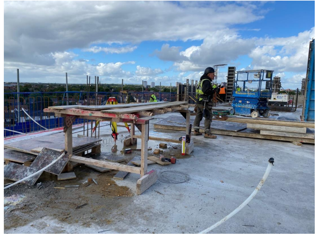
Block A concrete deck and column structure
