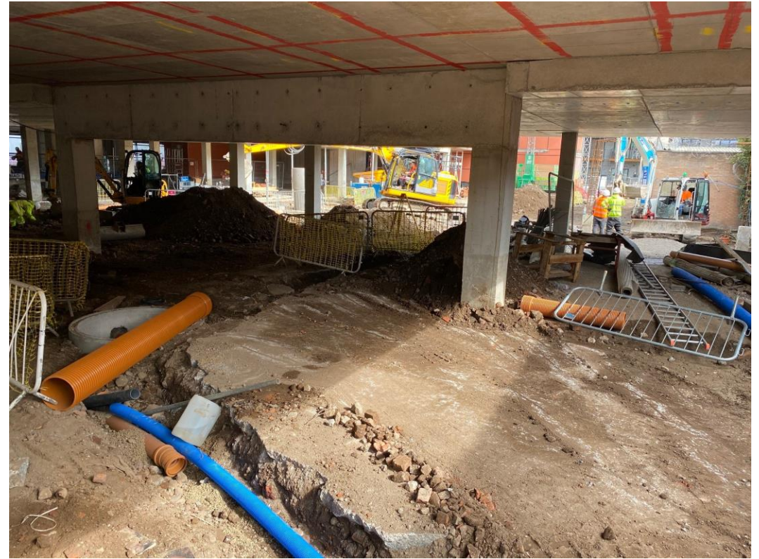
Block B drainage preparation
