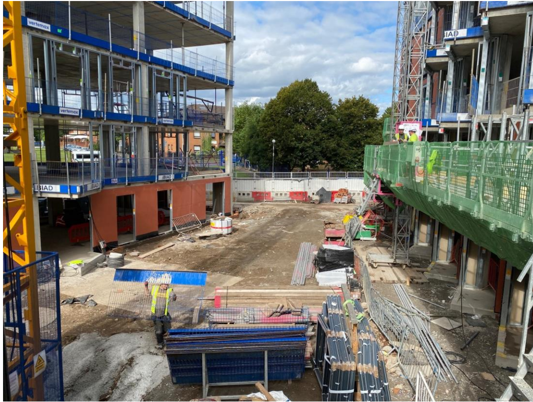
Block A SFS installation
