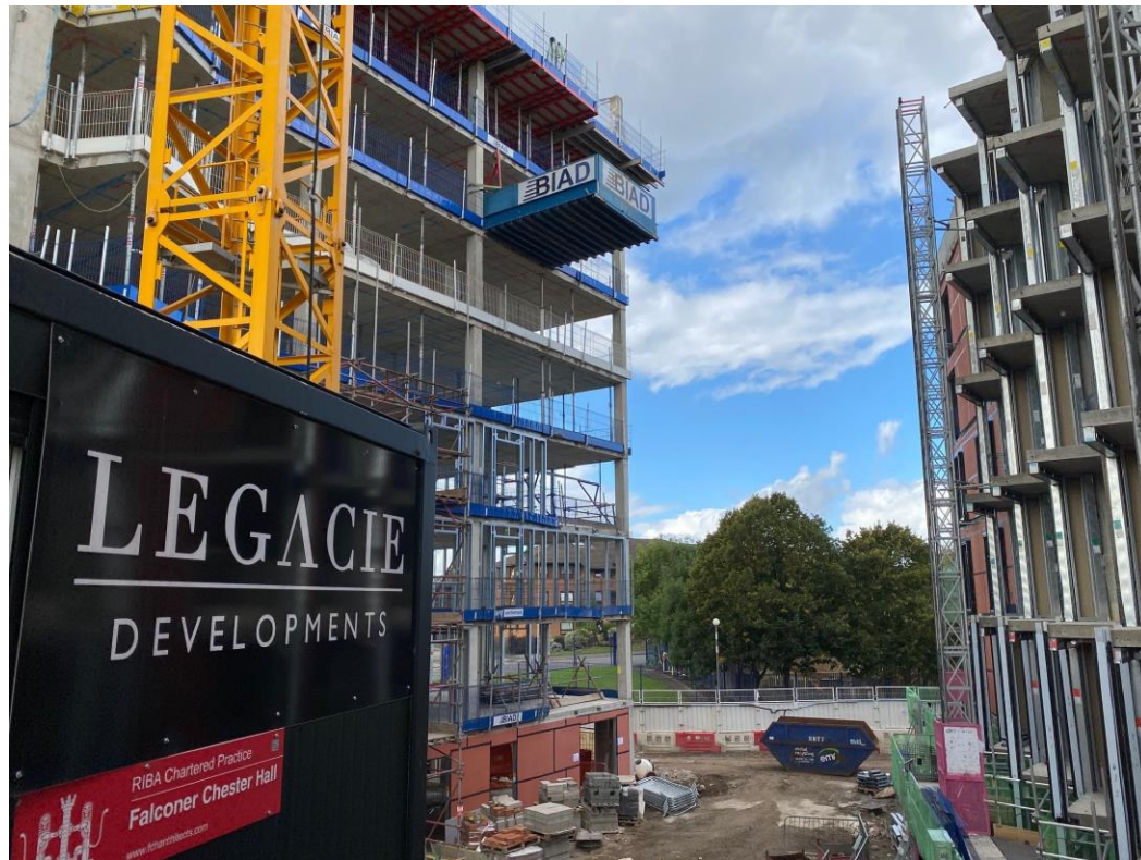
Block A & B SFS installation
