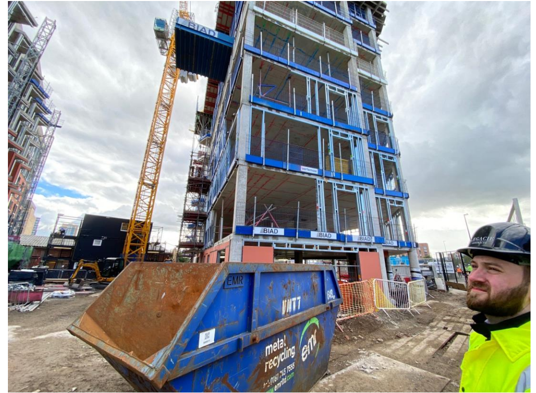
Block A SFS installation
