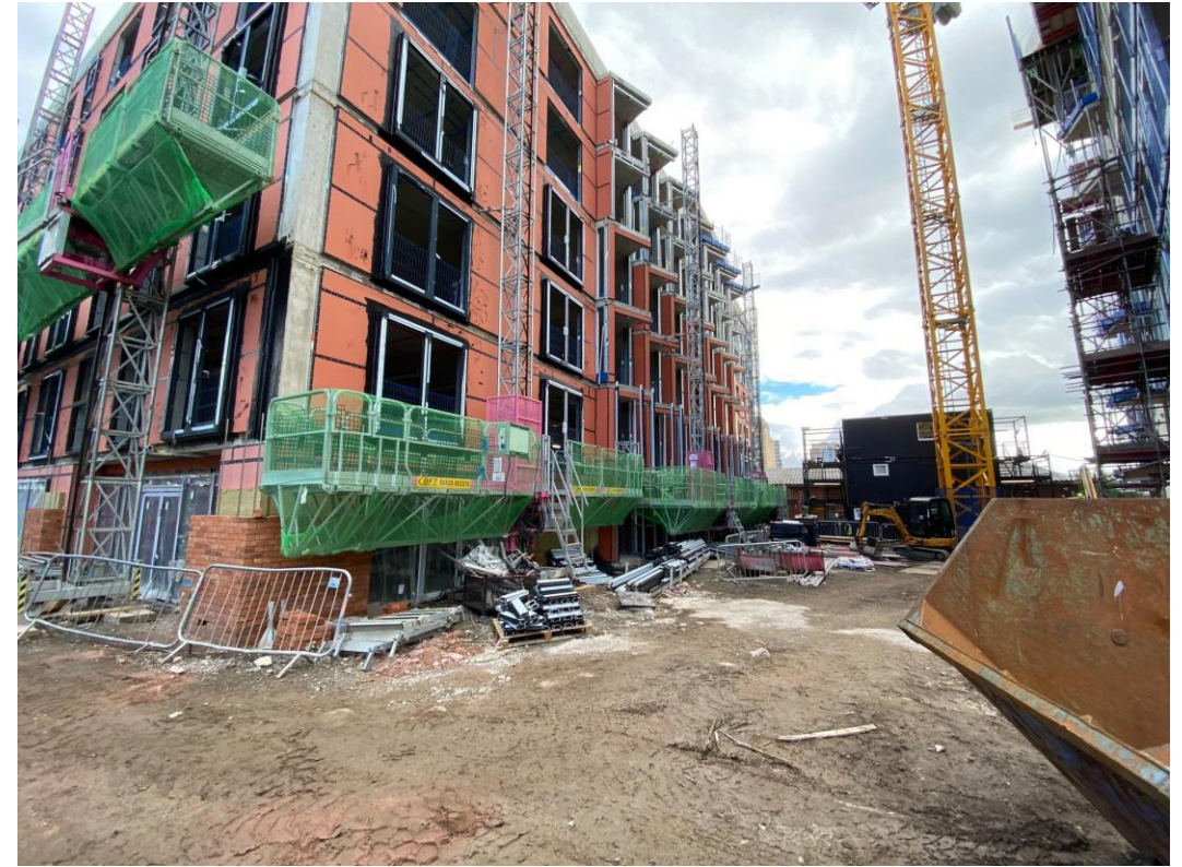
Block B SFS and weatherboarding
