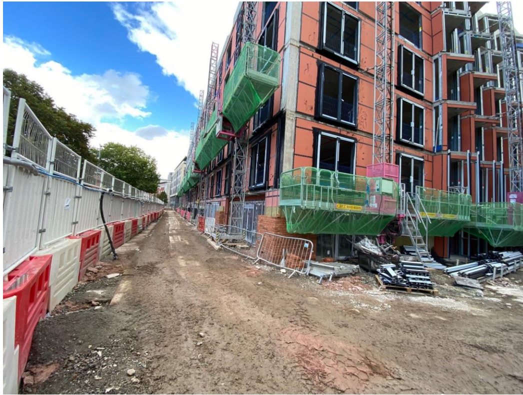
Block B SFS and weatherboarding
