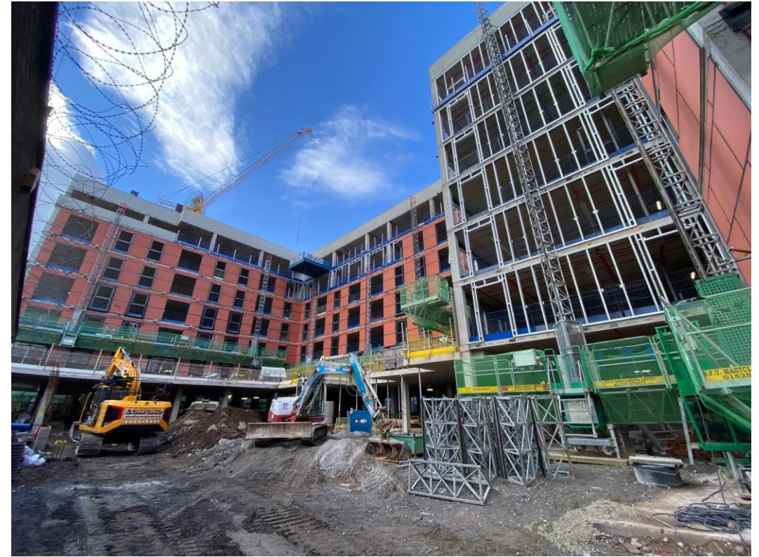
Block B SFS and weatherboarding
