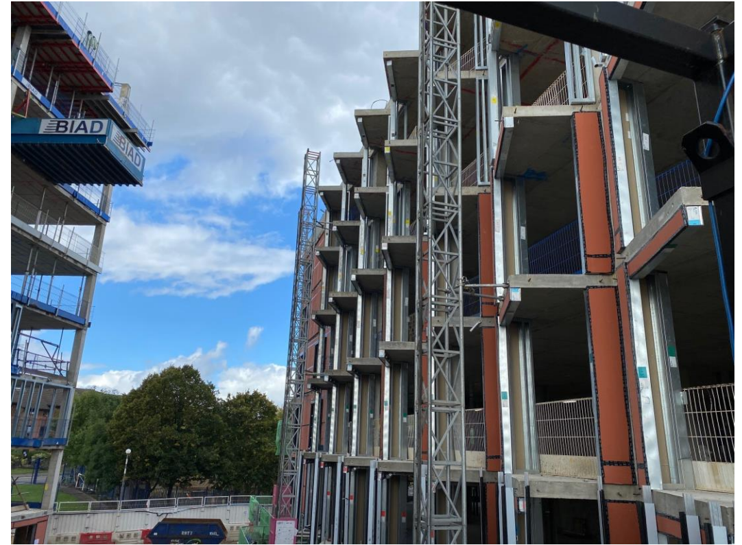
Block B SFS and weatherboarding
