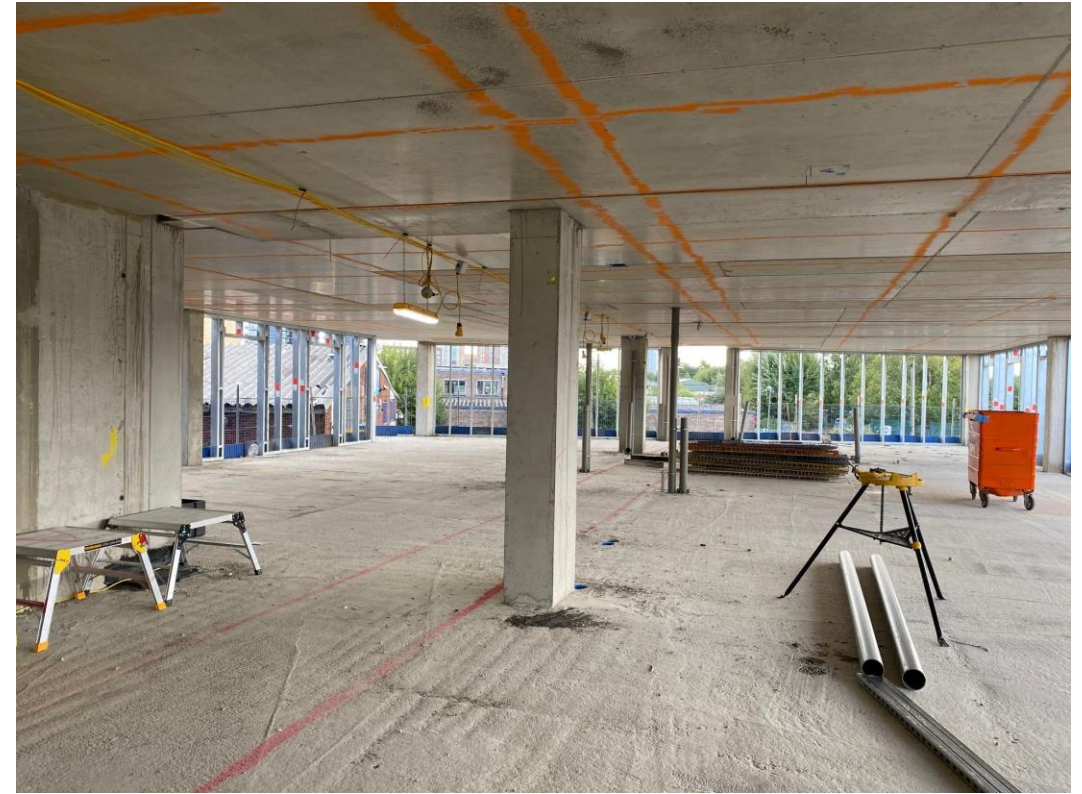
Block A upper floor SFS installation
