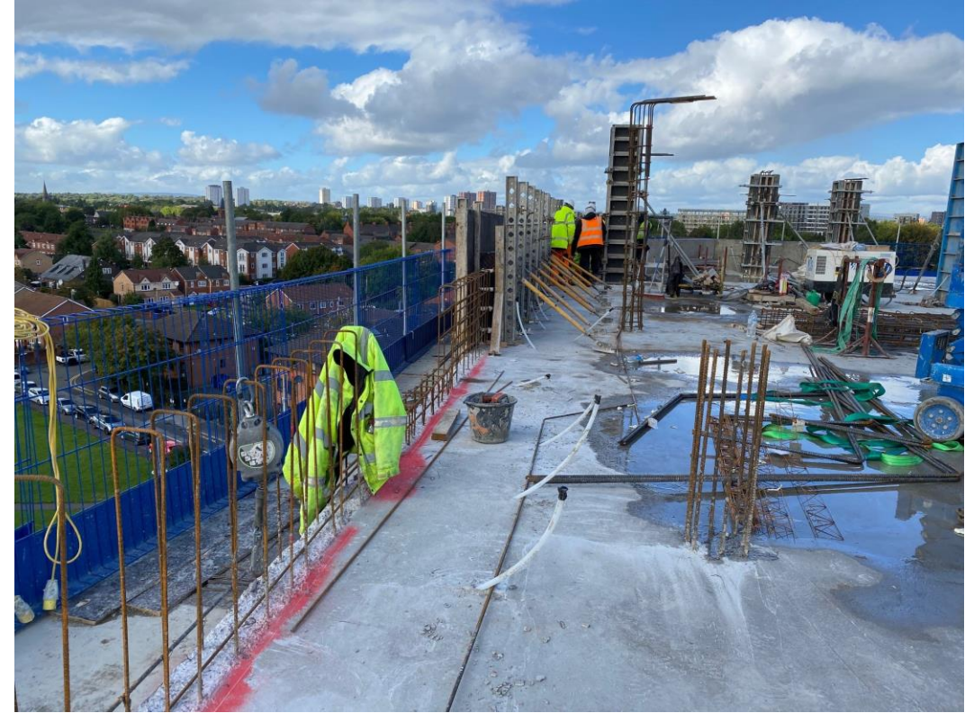
Block A concrete deck and column structure
