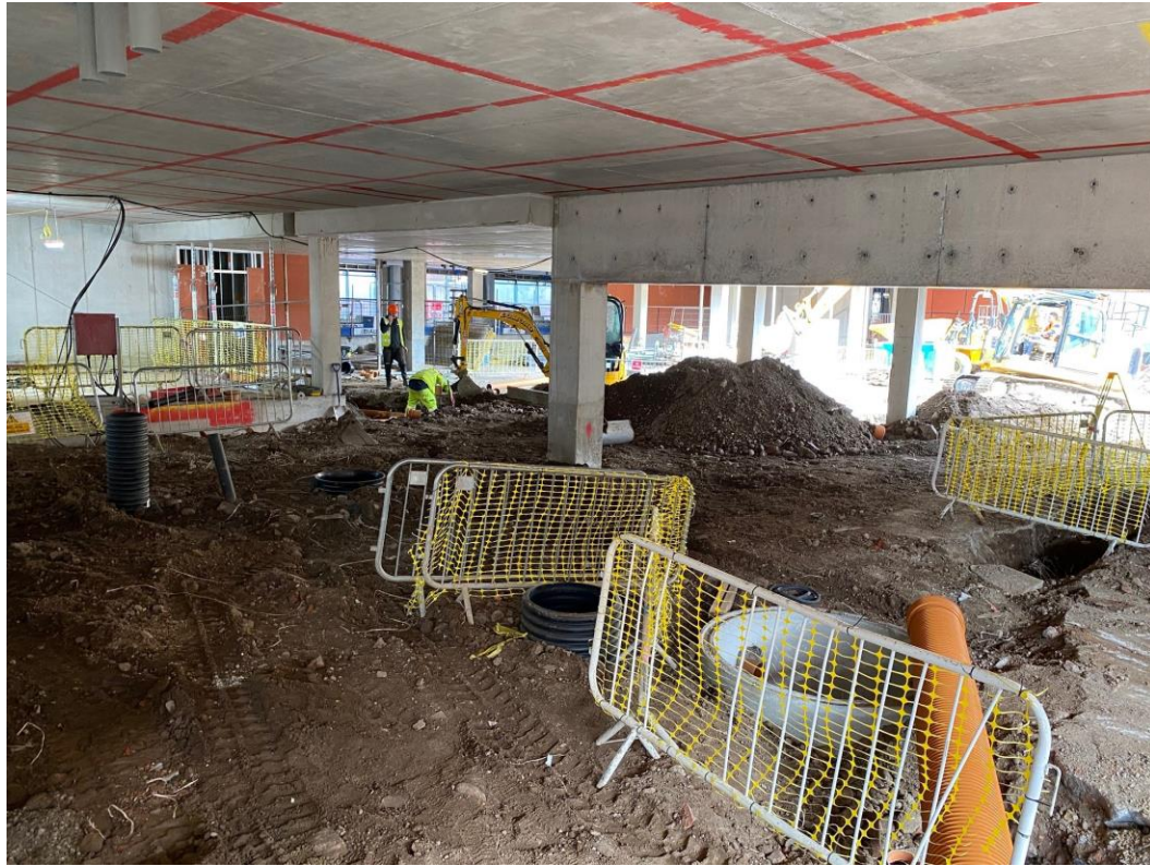
Block B drainage preparation
