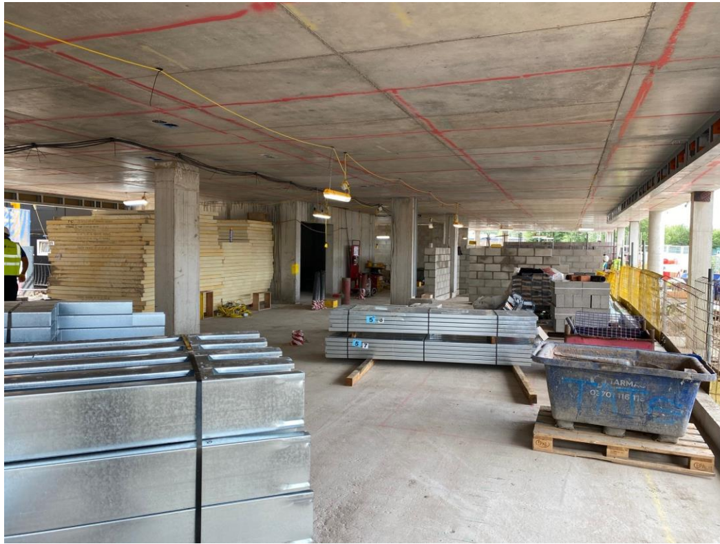
Block A ground floor blockwork
