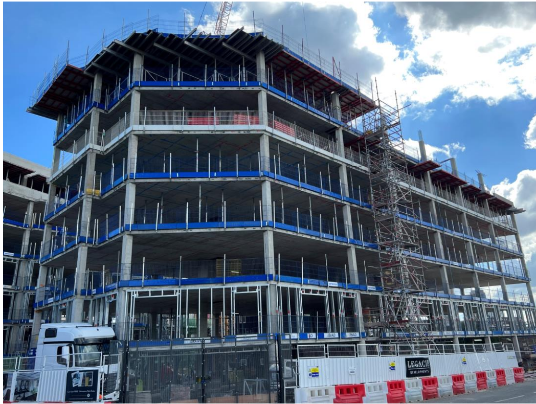
Ordsall Lane site view
