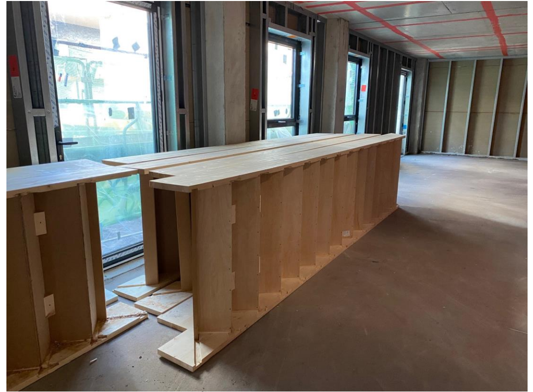
Block B timber staircase
