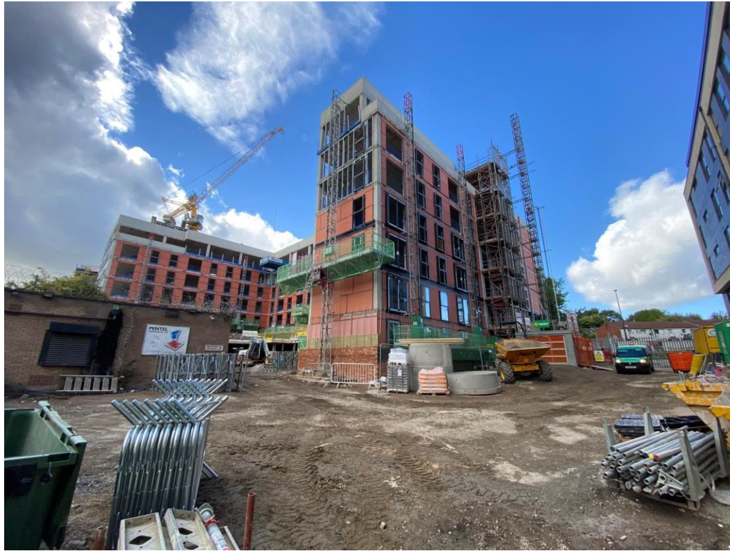
Block B SFS and weatherboarding
