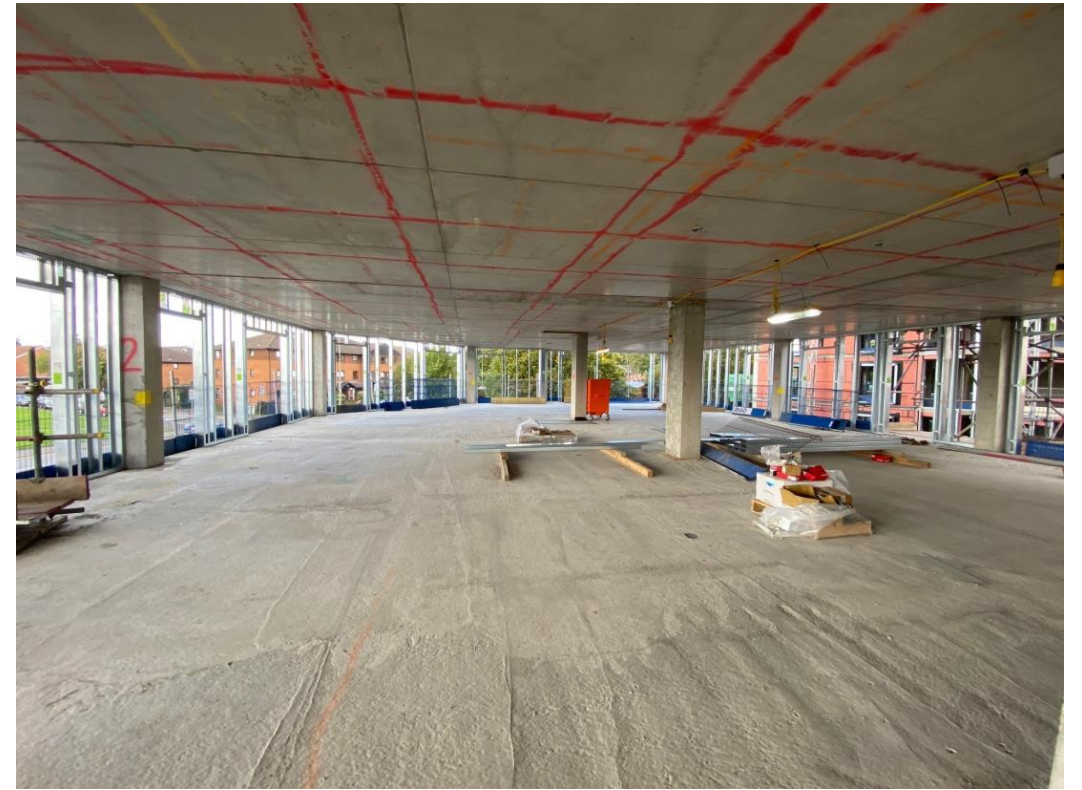
Block A upper floor SFS installation
