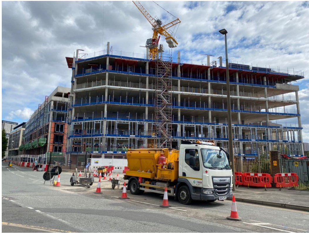
Ordsall Lane site view
