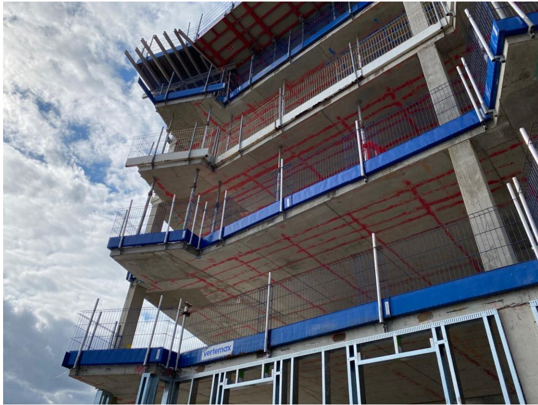
Block A concrete framework
