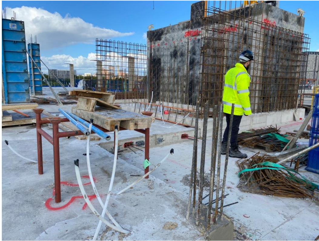
Block A concrete deck and column structure
