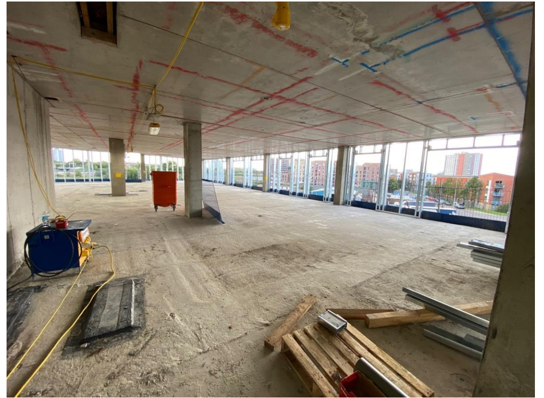
Block A upper floor SFS installation
