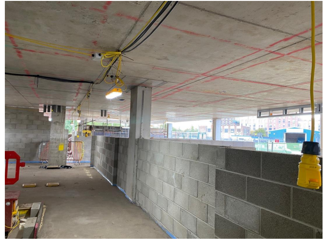
Block A ground floor slab preparation
