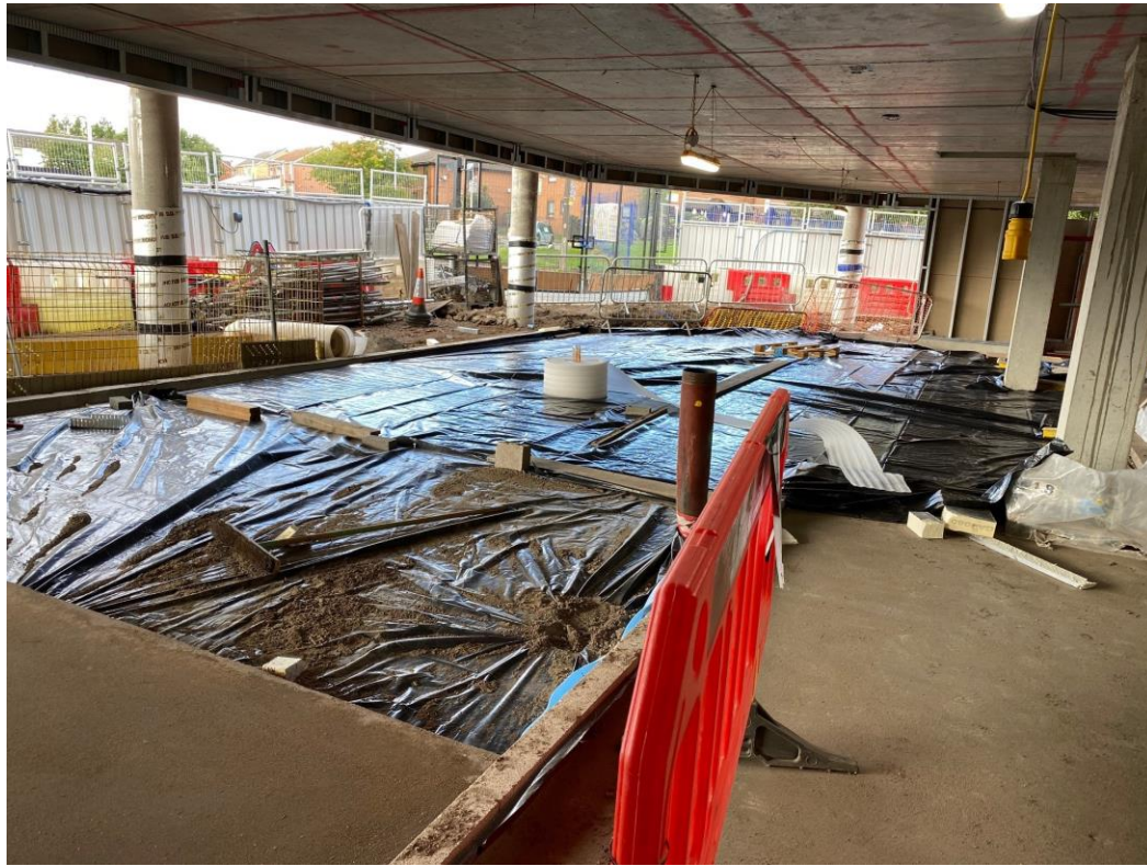
Block A ground floor screed
