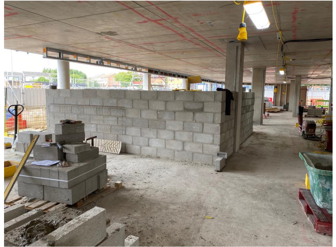
Block A ground floor blockwork
