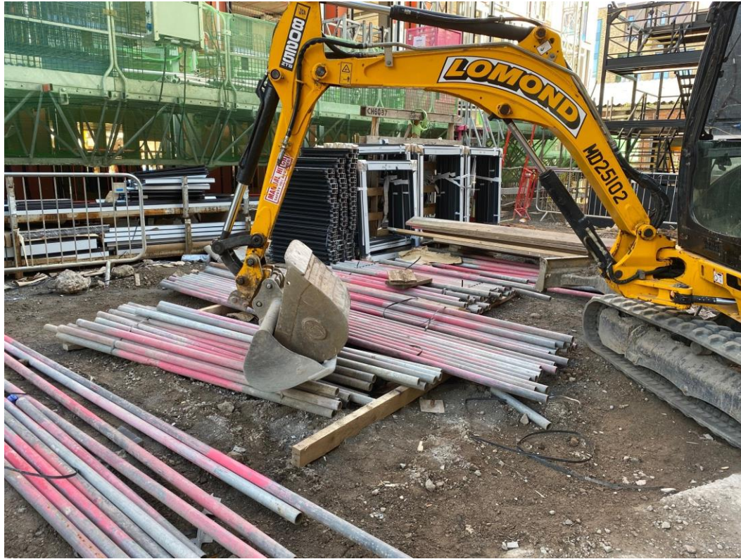
Block B curtain walling
