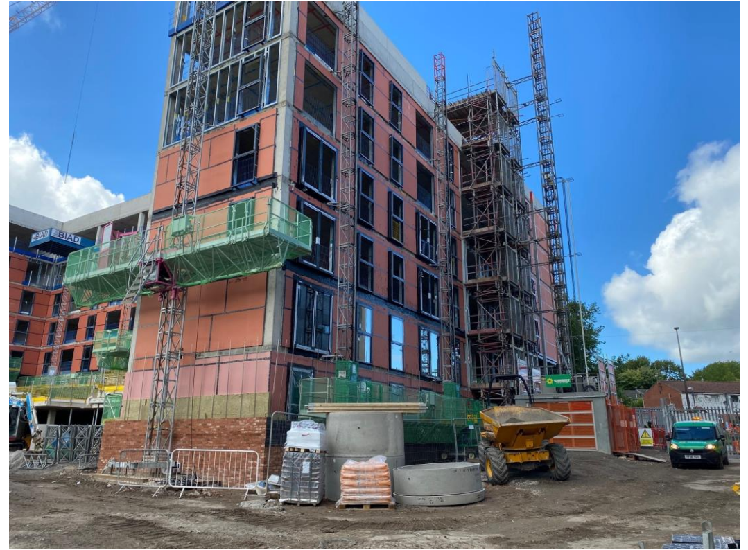
Block B SFS and weatherboarding
