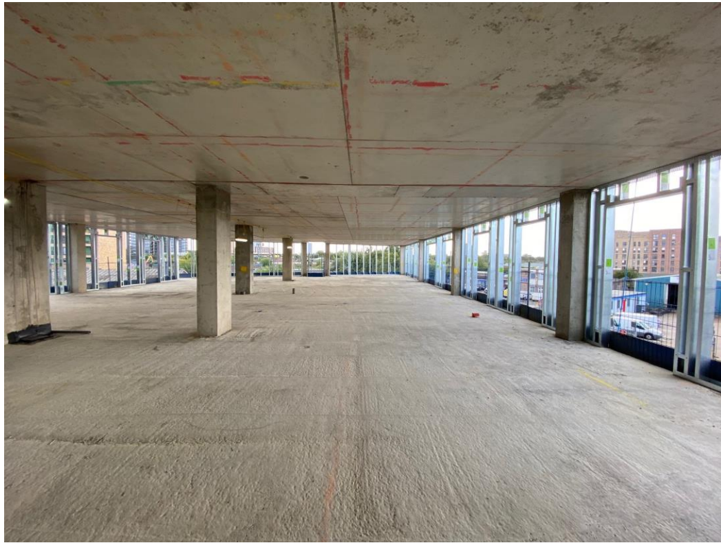
Block A upper floor SFS installation
