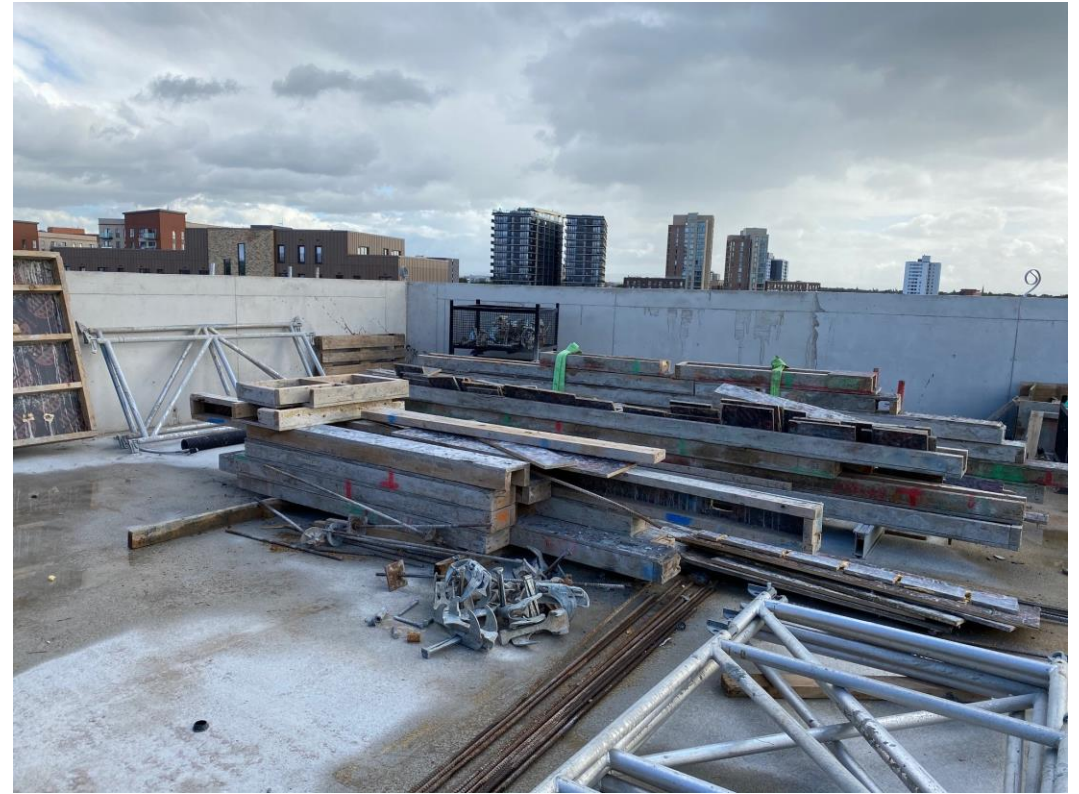
Block B Roof and parapet
