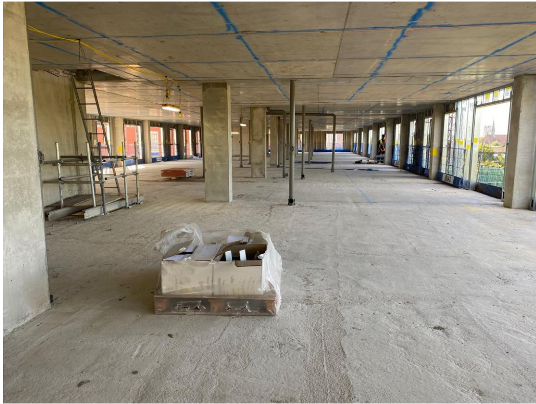
Block A upper floor SFS installation
