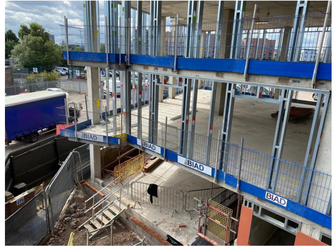
Block A SFS installation
