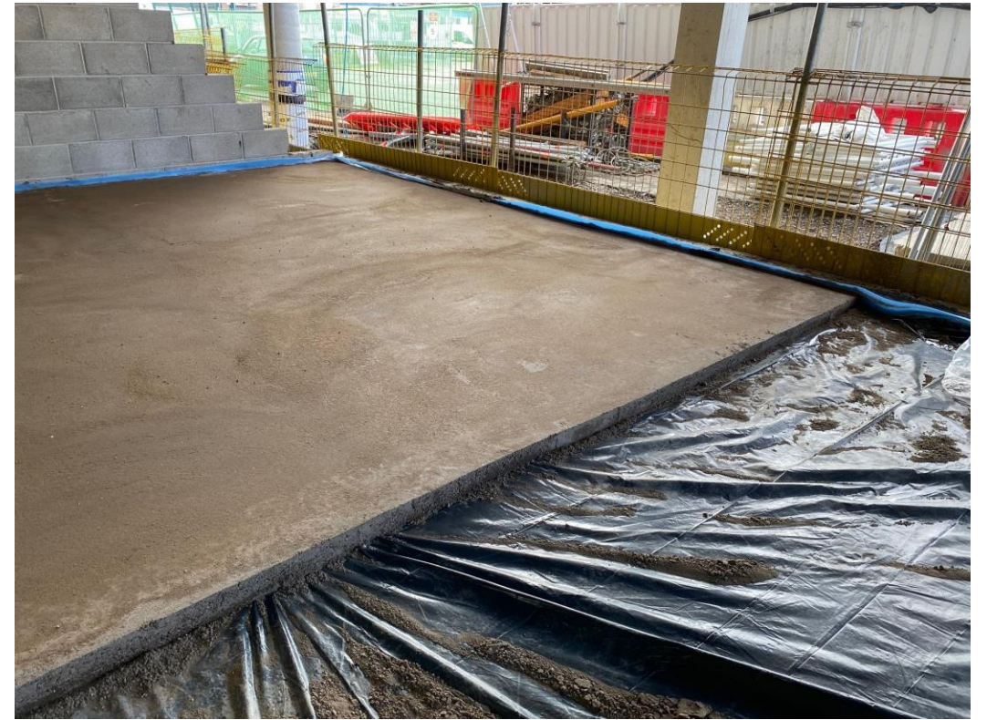
Block A ground floor screed preparation
