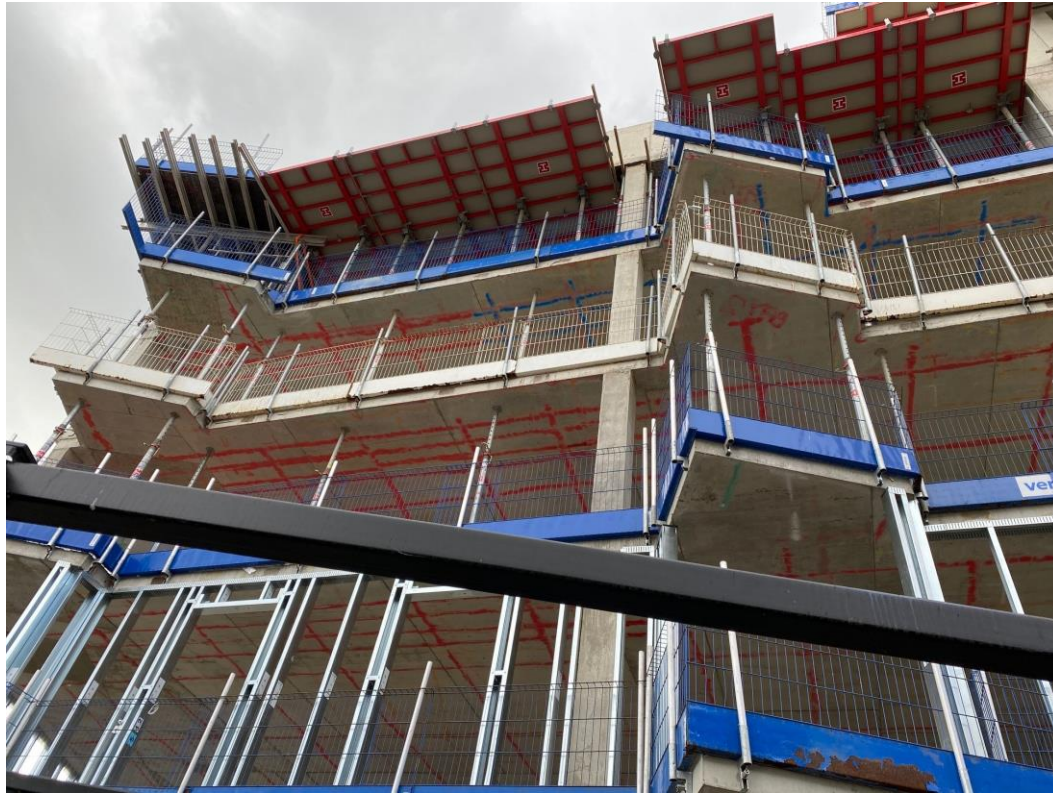
Block A SFS installation
