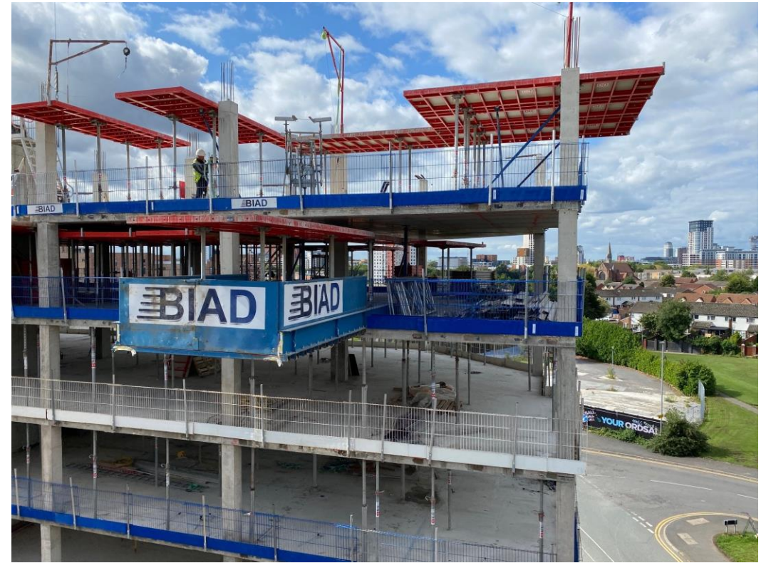
Block A concrete framework
