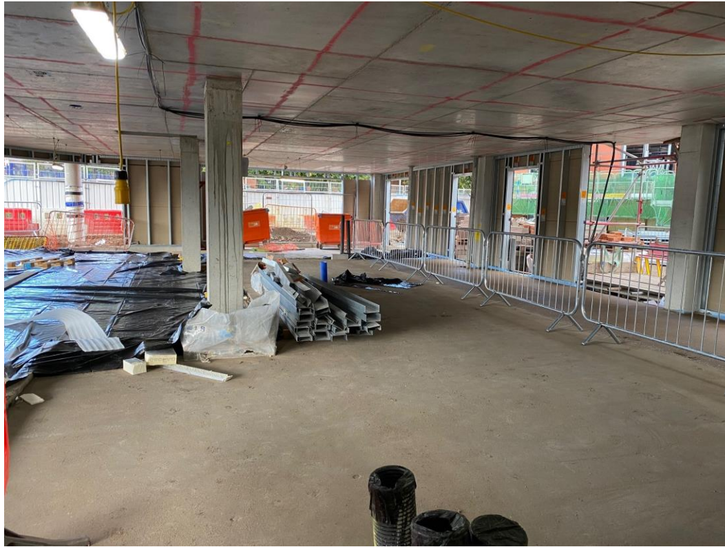
Block A ground floor slab preparation
