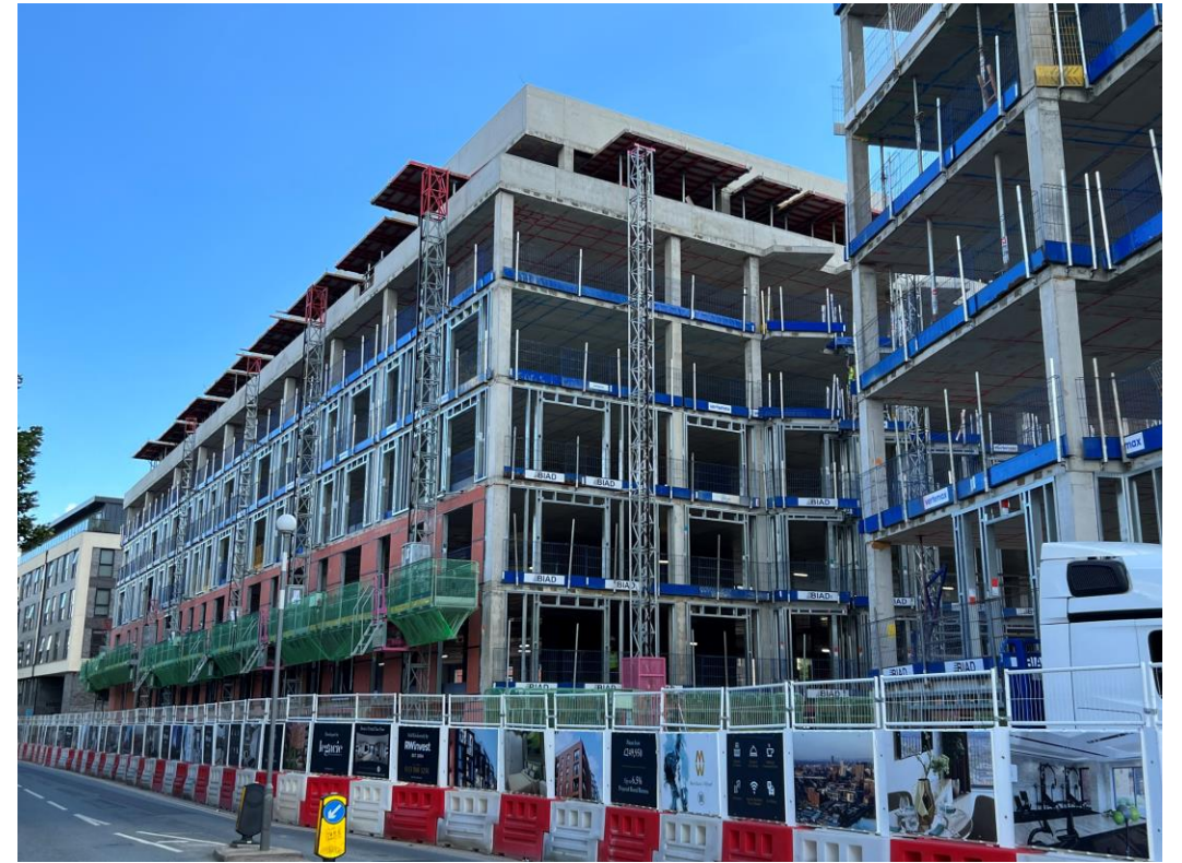
Ordsall Lane site view
