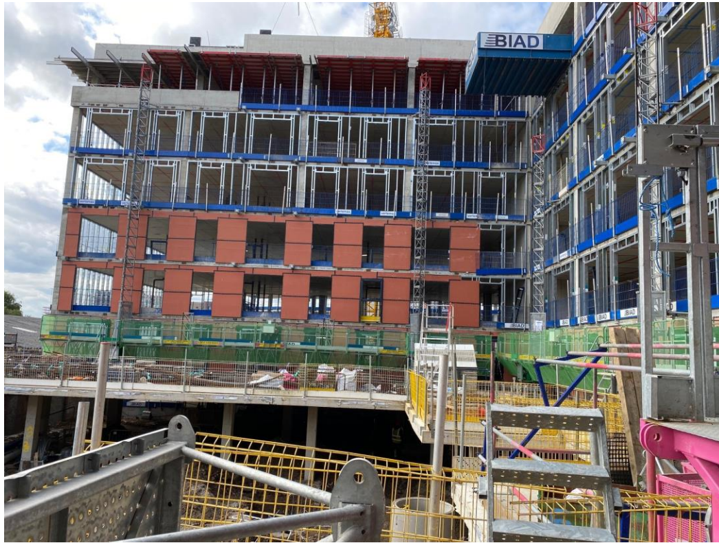
Block B SFS and weatherboarding
