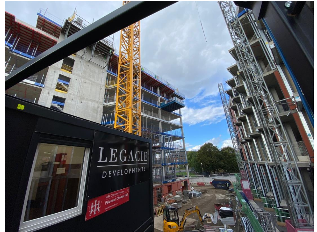
Block A & B SFS installation
