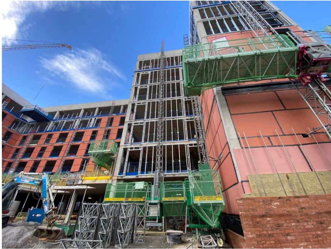
Block B SFS and weatherboarding
