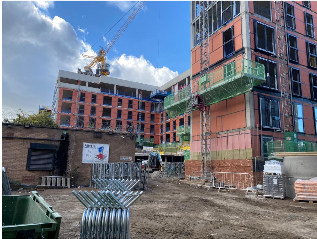
Block B SFS and weatherboarding
