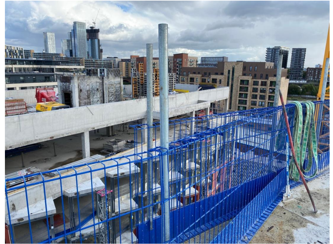
Block B Roof and parapet
