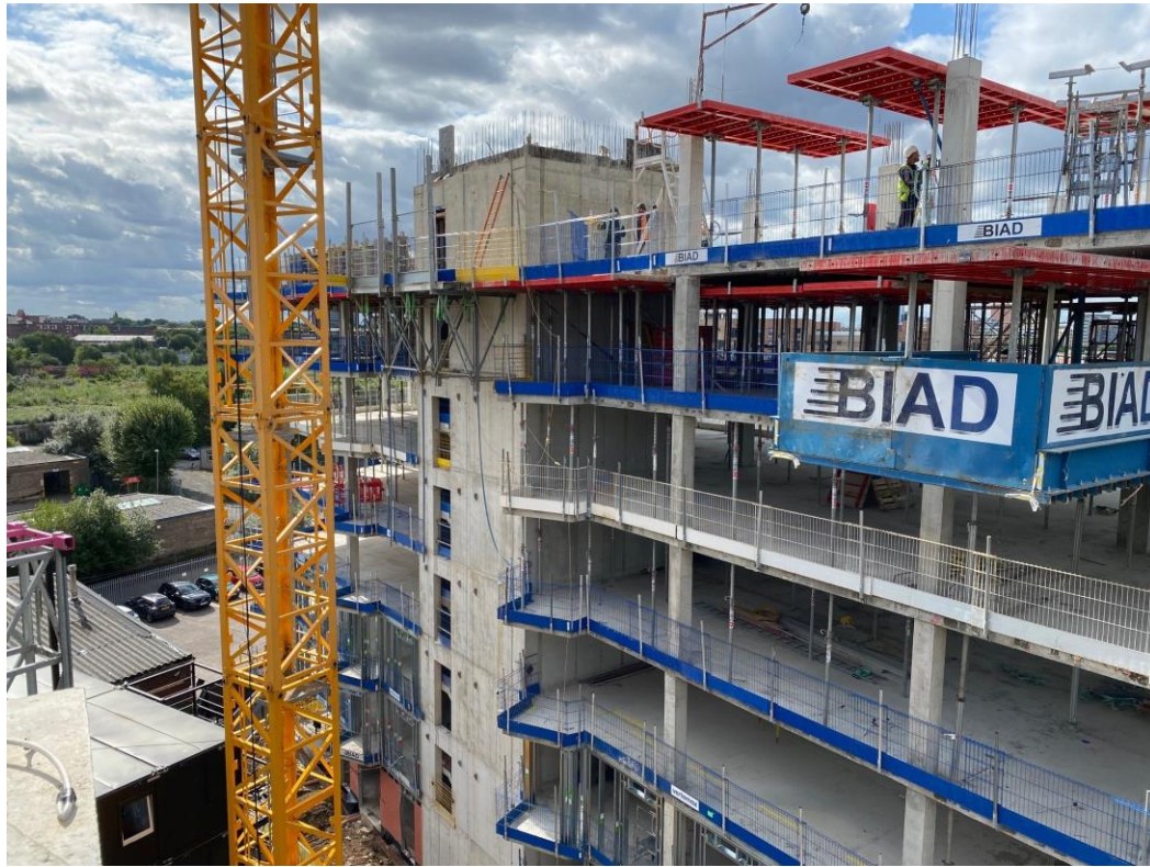
Block A concrete framework
