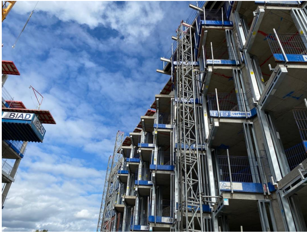
Block B concrete framework
