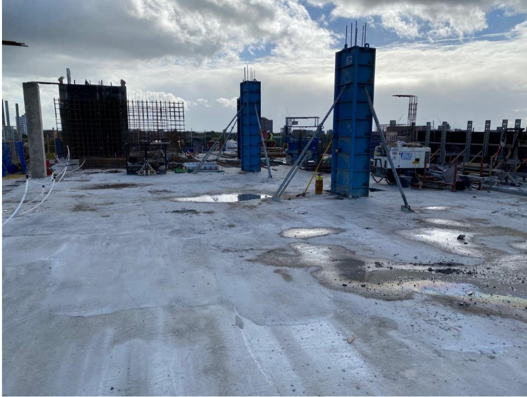
Block A concrete deck and column structure
