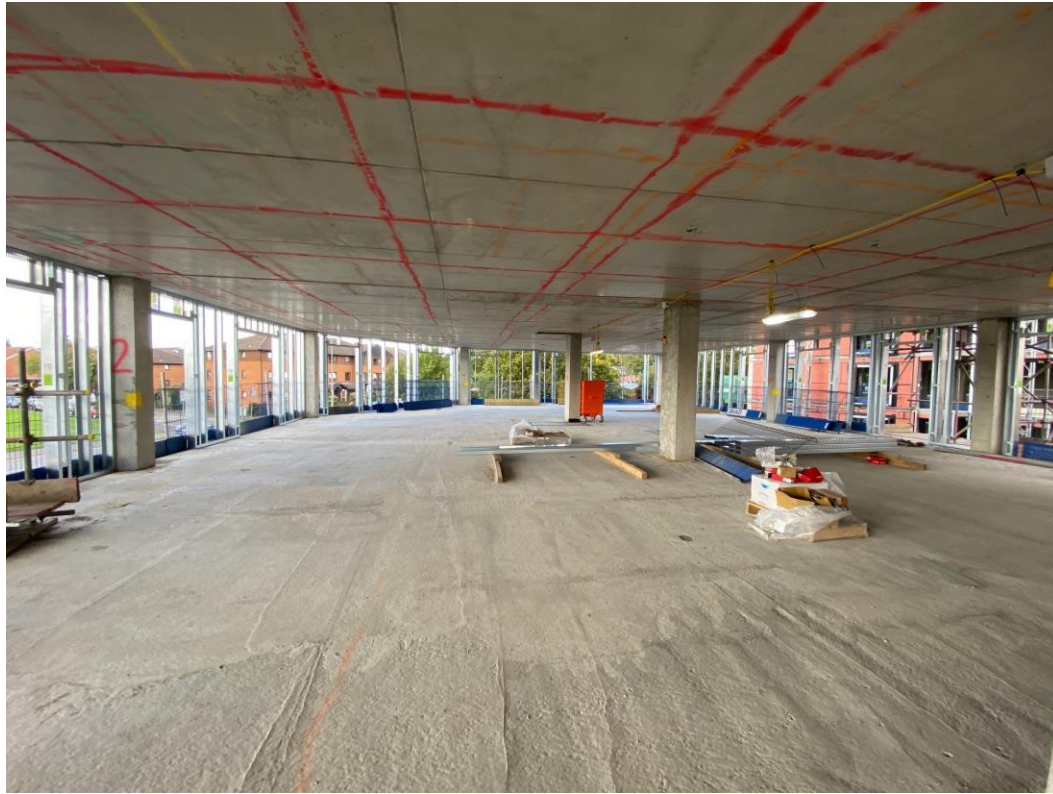
Block A upper floor SFS installation
