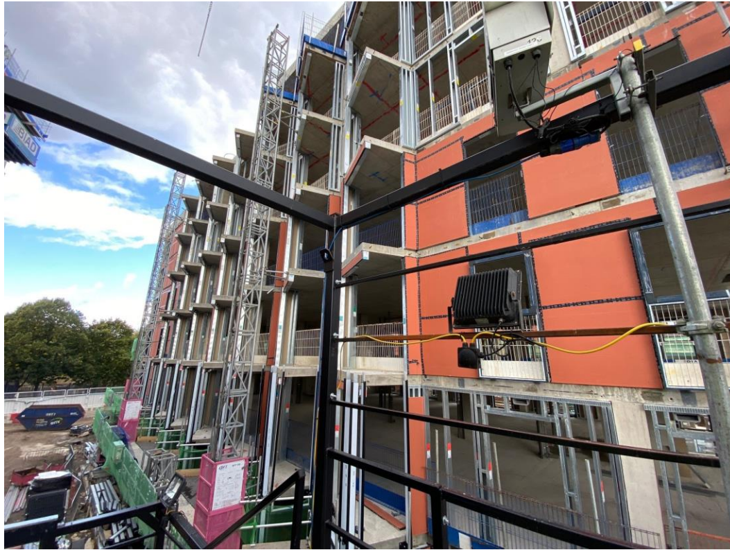
Block B SFS and weatherboarding
