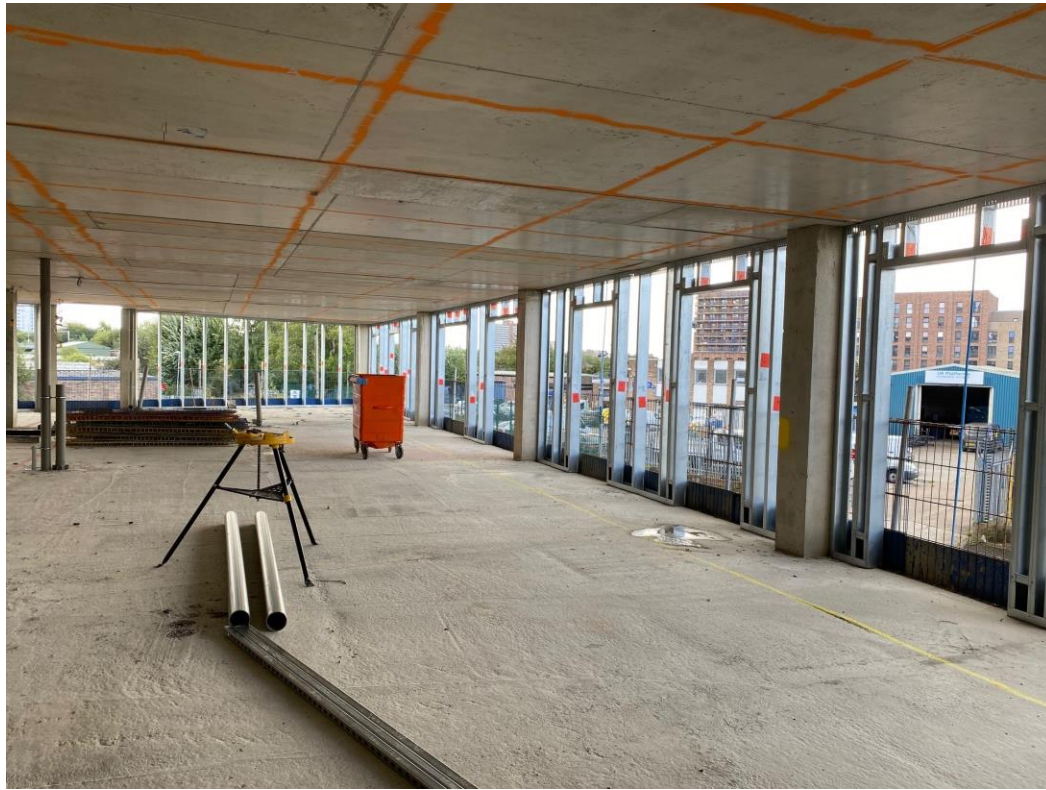
Block A upper floor SFS installation
