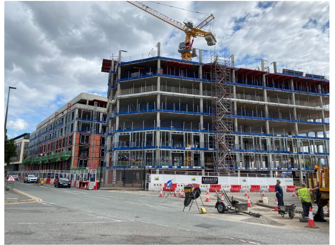
Ordsall Lane site view
