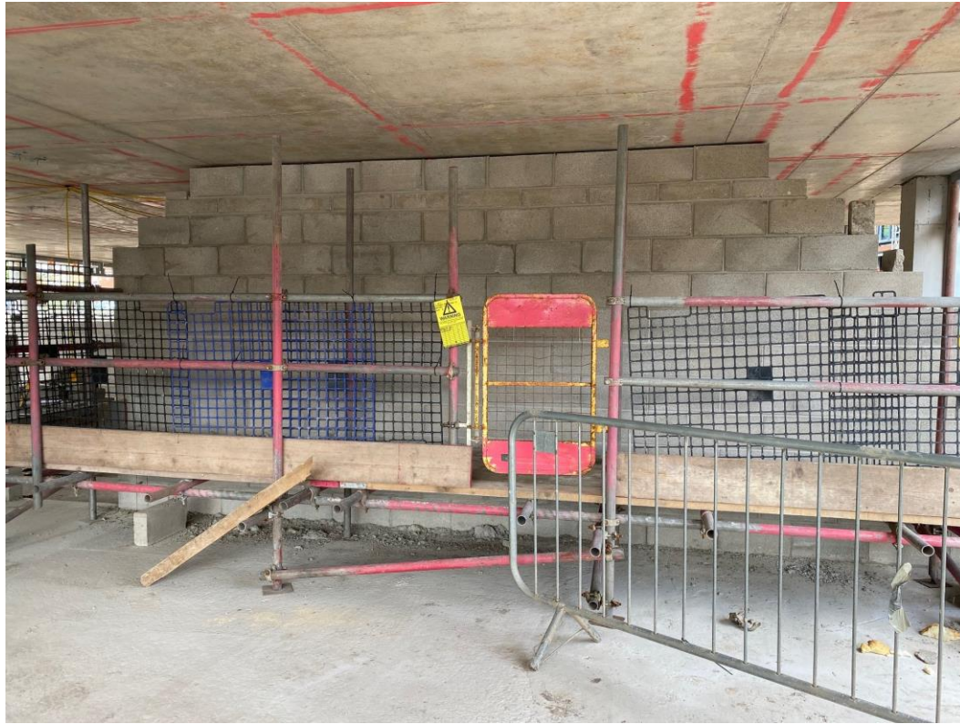
Block A ground floor blockwork
