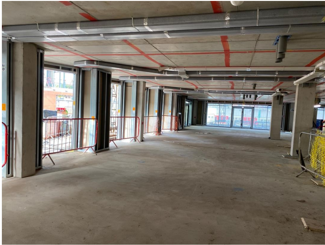
Block B above ground drainage & mechanical ducting installation
