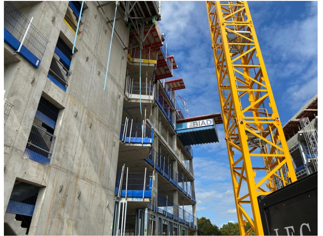
Block A concrete framework
