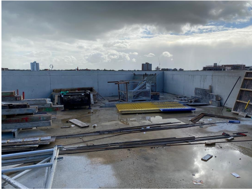
Block B Roof and parapet
