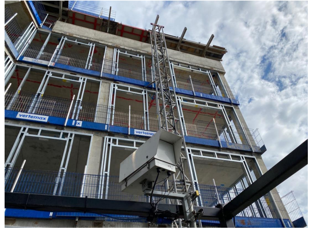
Block B SFS installation
