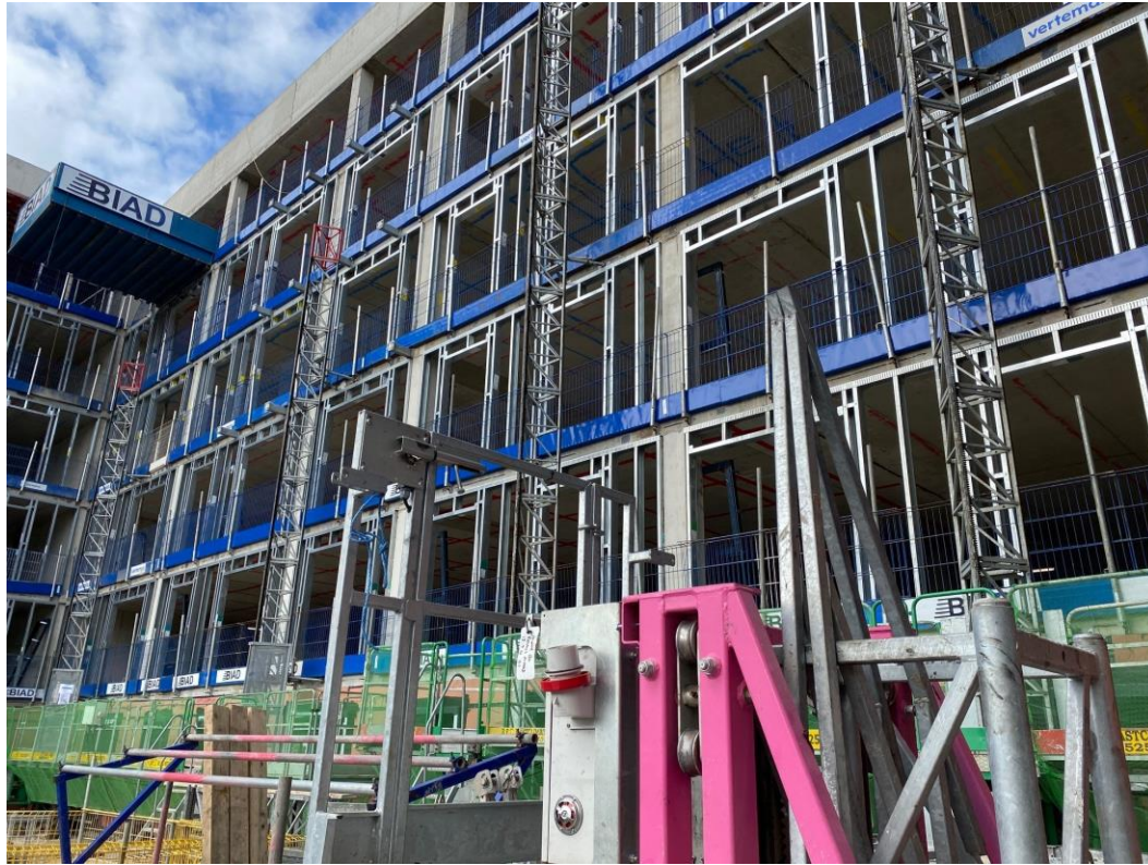
Block B SFS installation
