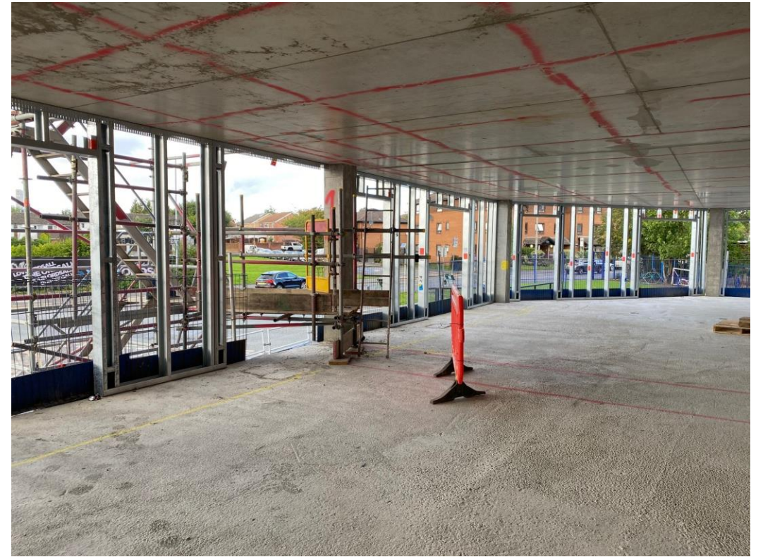
Block A upper floor SFS installation
