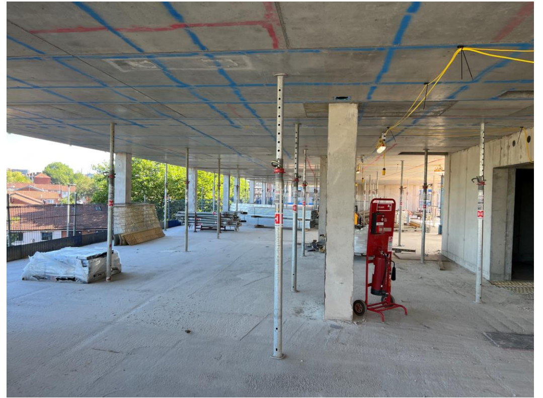
Block B Third Floor concrete structure
