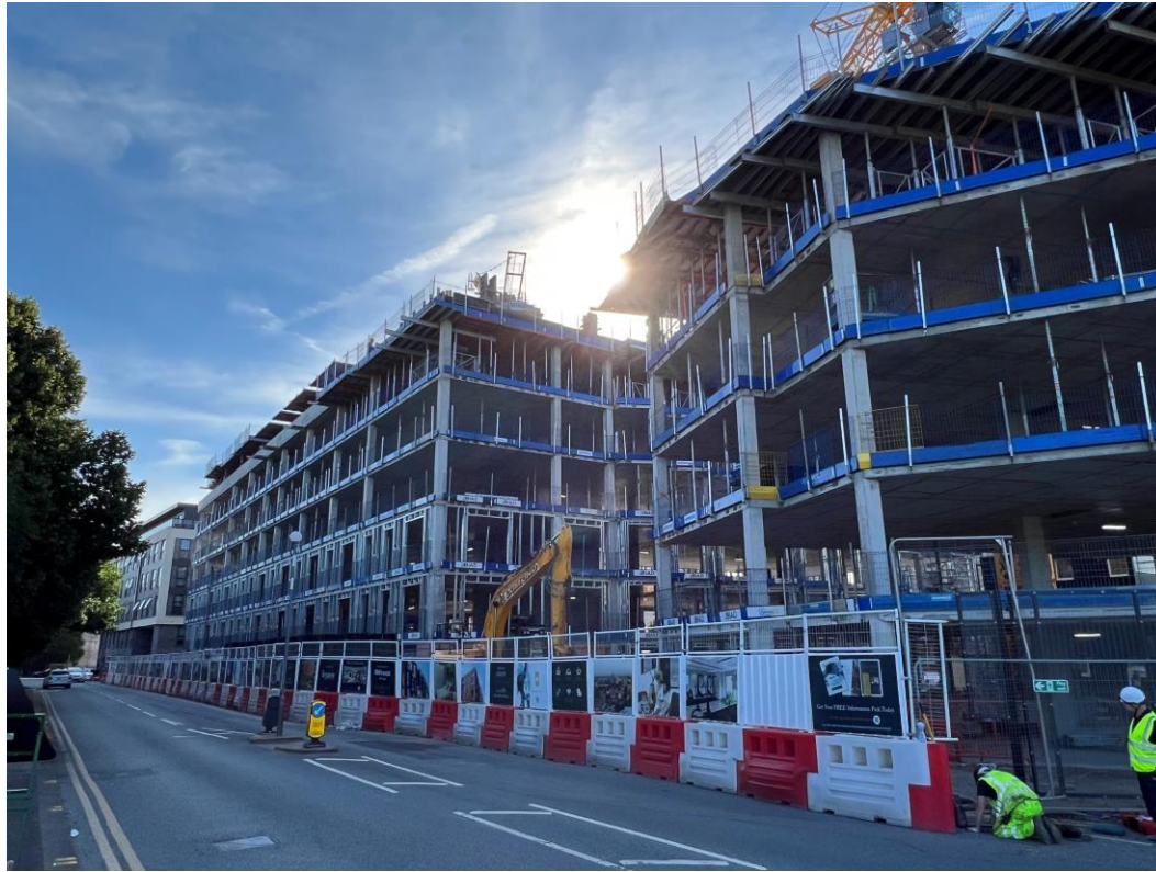
Ordsall Lane site view
