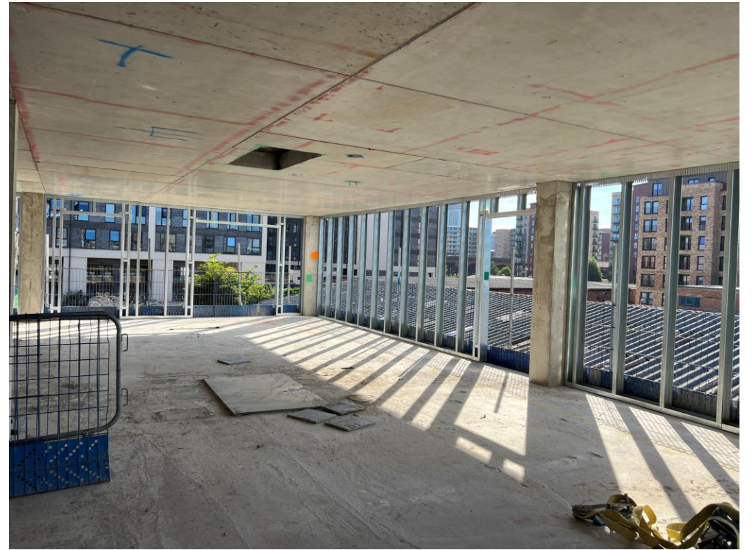
Block B Second Floor concrete structure
