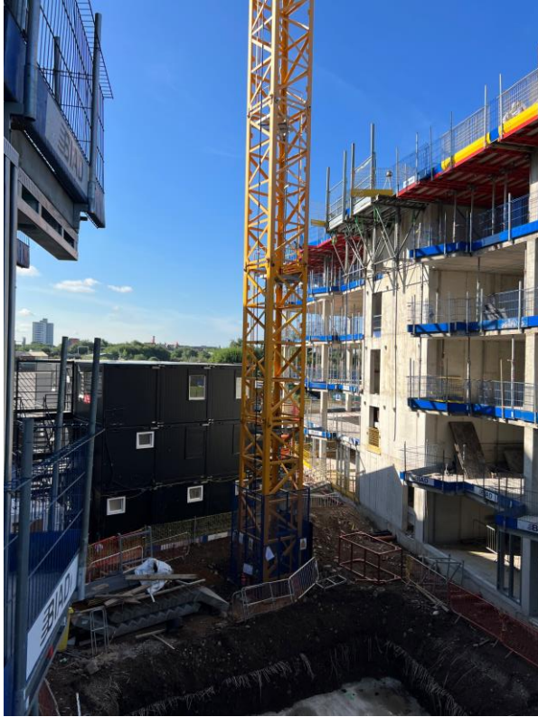
Block A concrete framework
