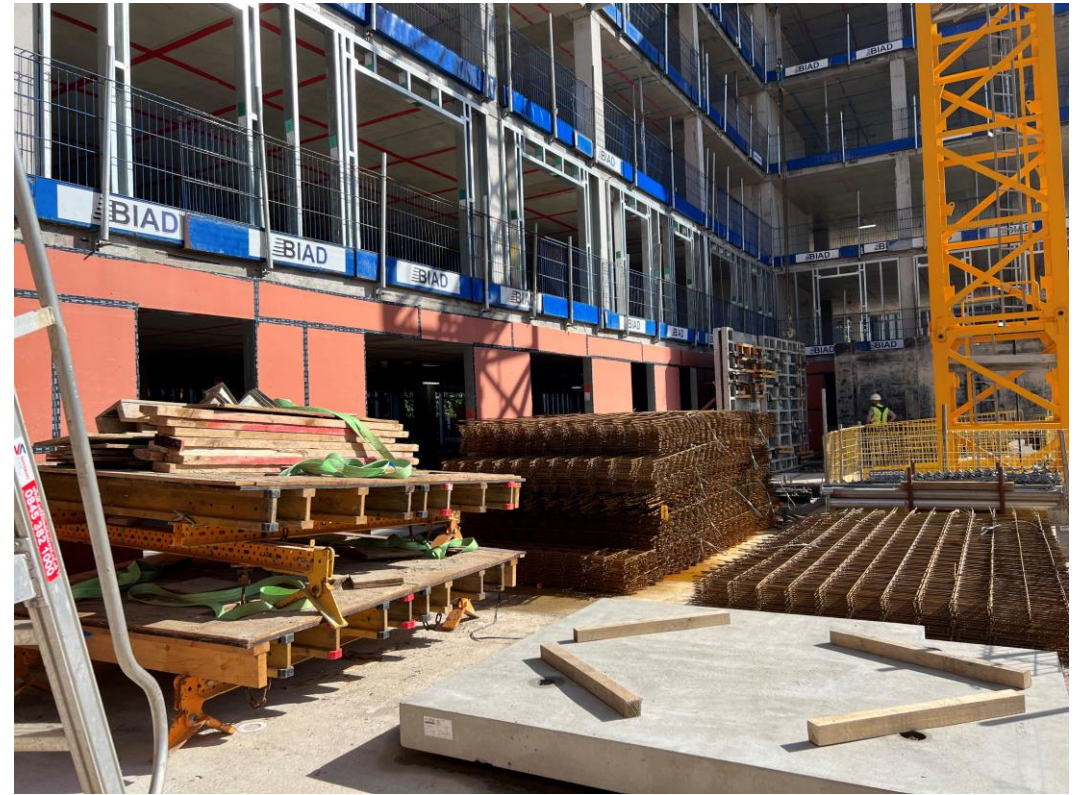
Block B structure and weatherboarding
