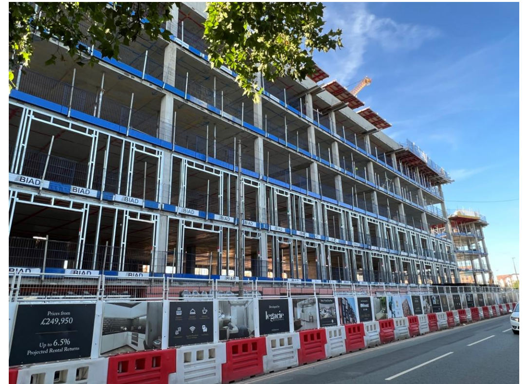
Ordsall Lane site view
