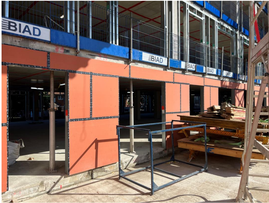
Block B structure and weatherboarding
