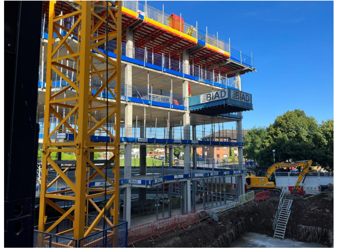
Block A concrete framework
