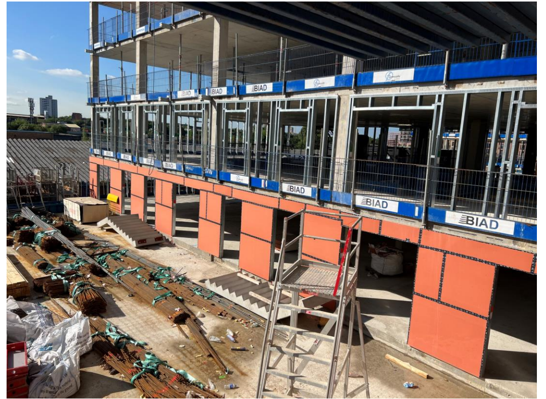
Block B structure and weatherboarding
