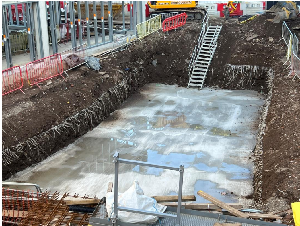
Block A & B attenuation drainage preparation
