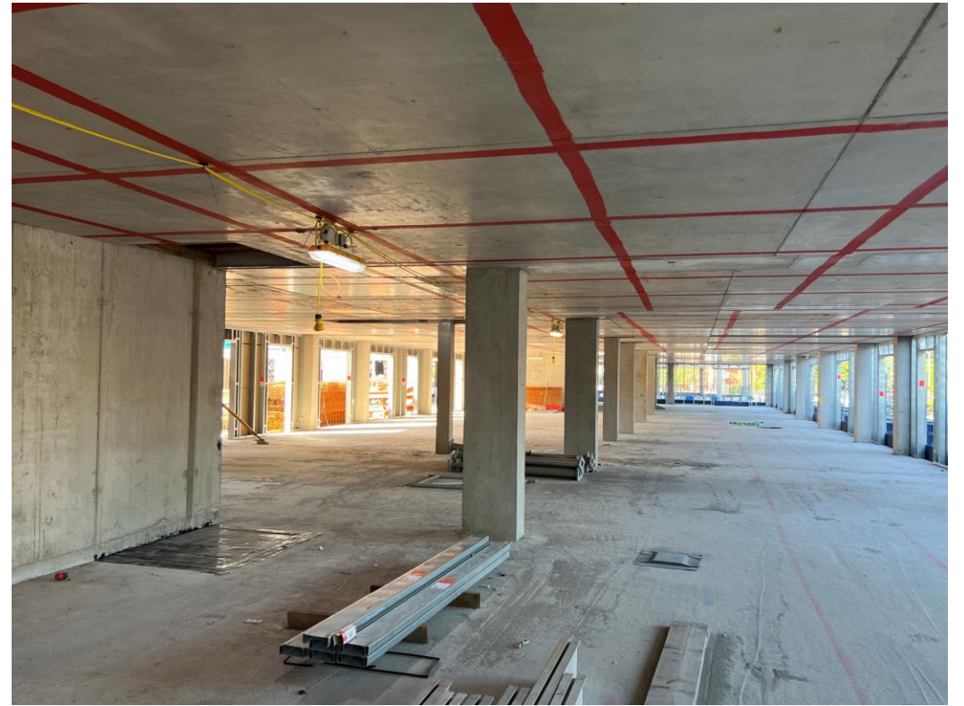
Block B First Floor concrete structure
