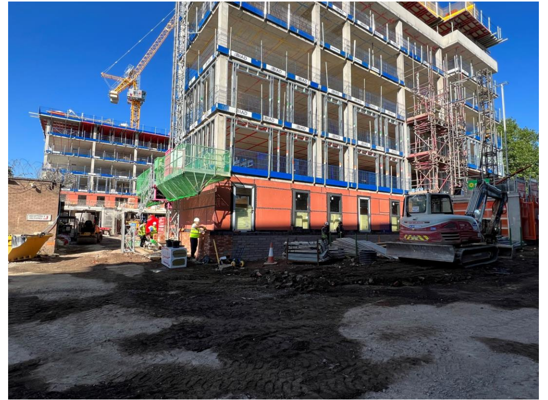
Block B Facing brickwork
