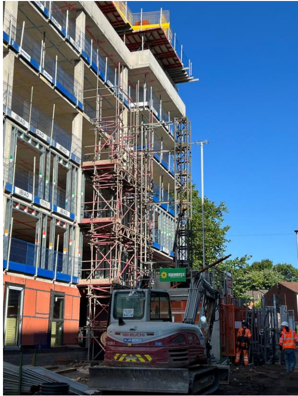
Block B hoist access installed
