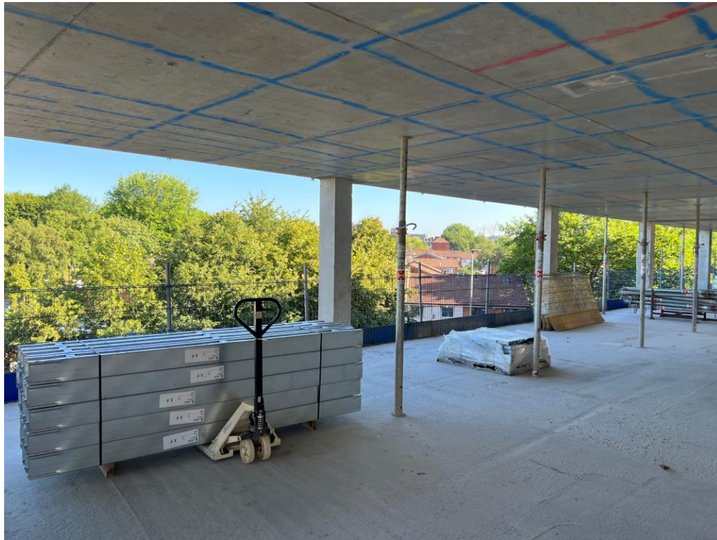
Block B Third Floor SFS materials
