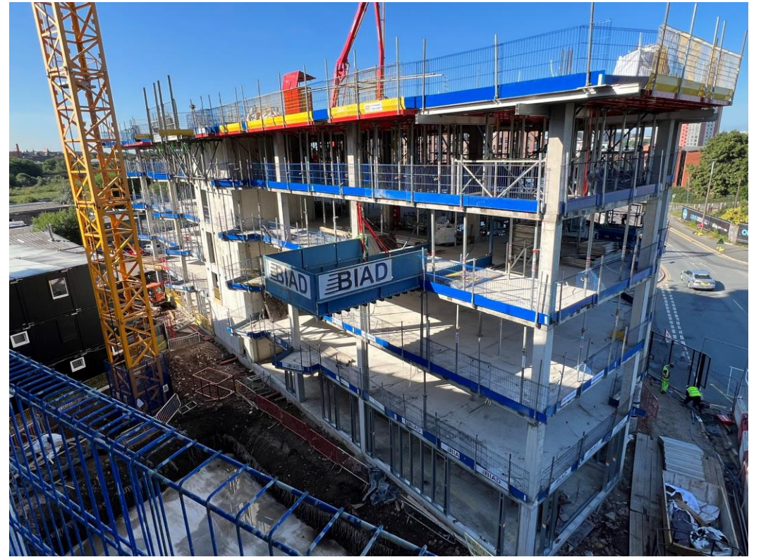
Block A concrete framework
