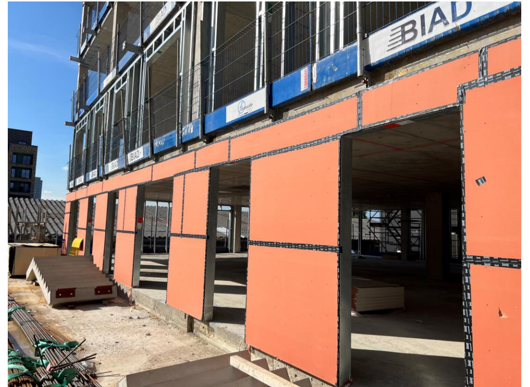
Block B structure and weatherboarding
