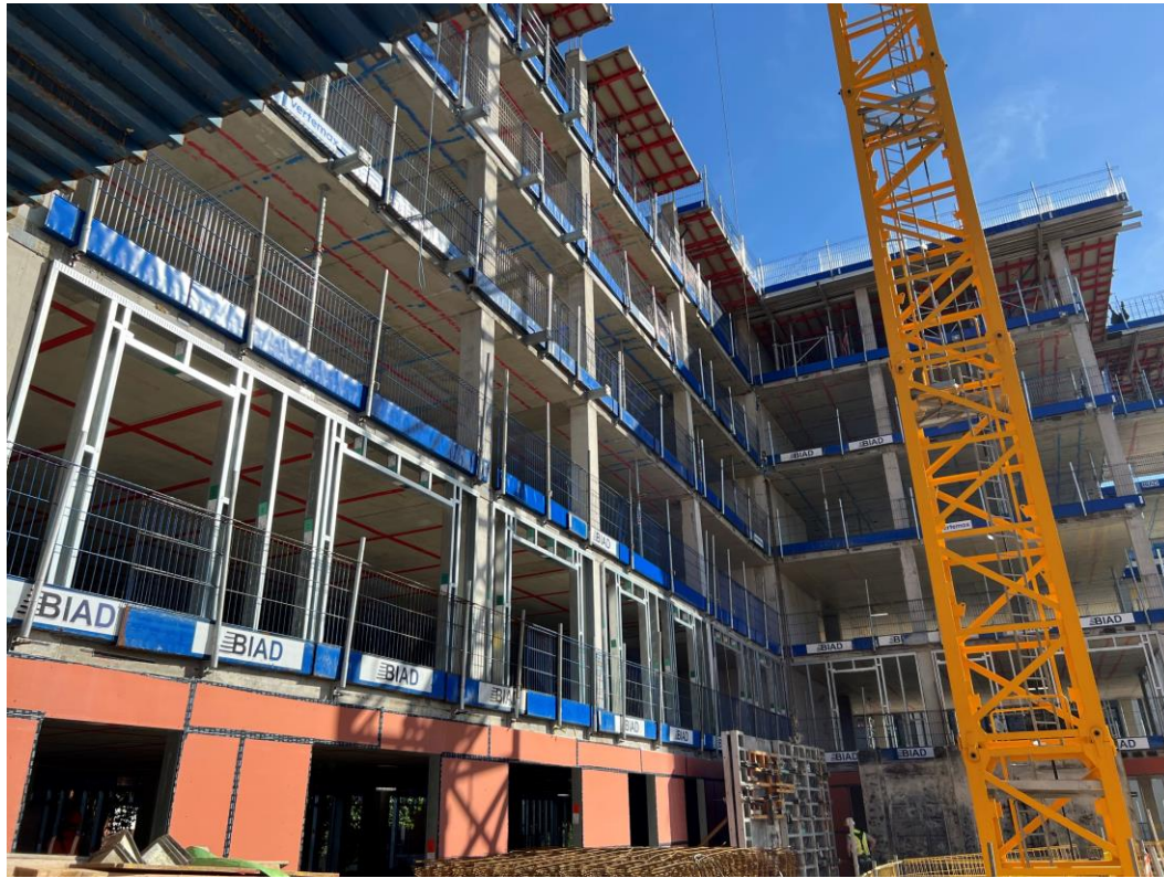
Block B structure and weatherboarding
