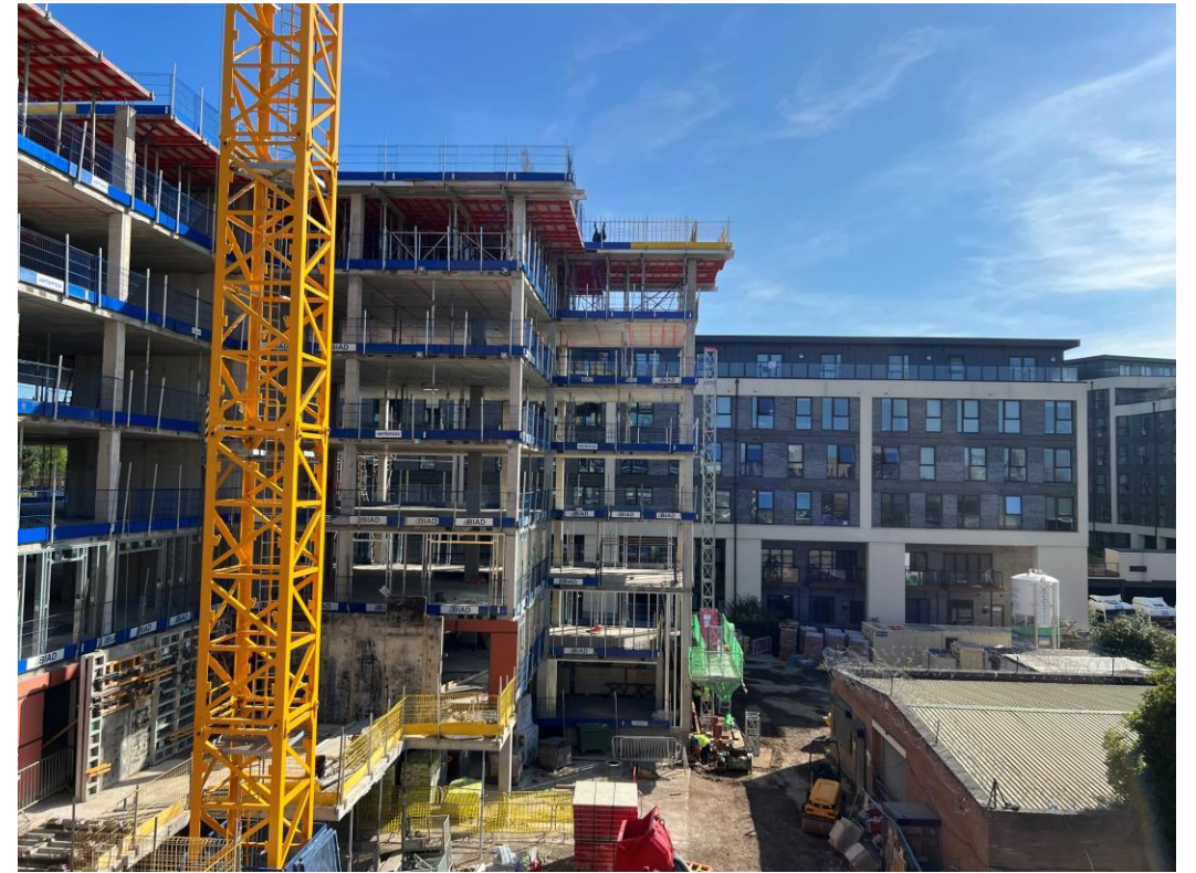
Block B structure and weatherboarding
