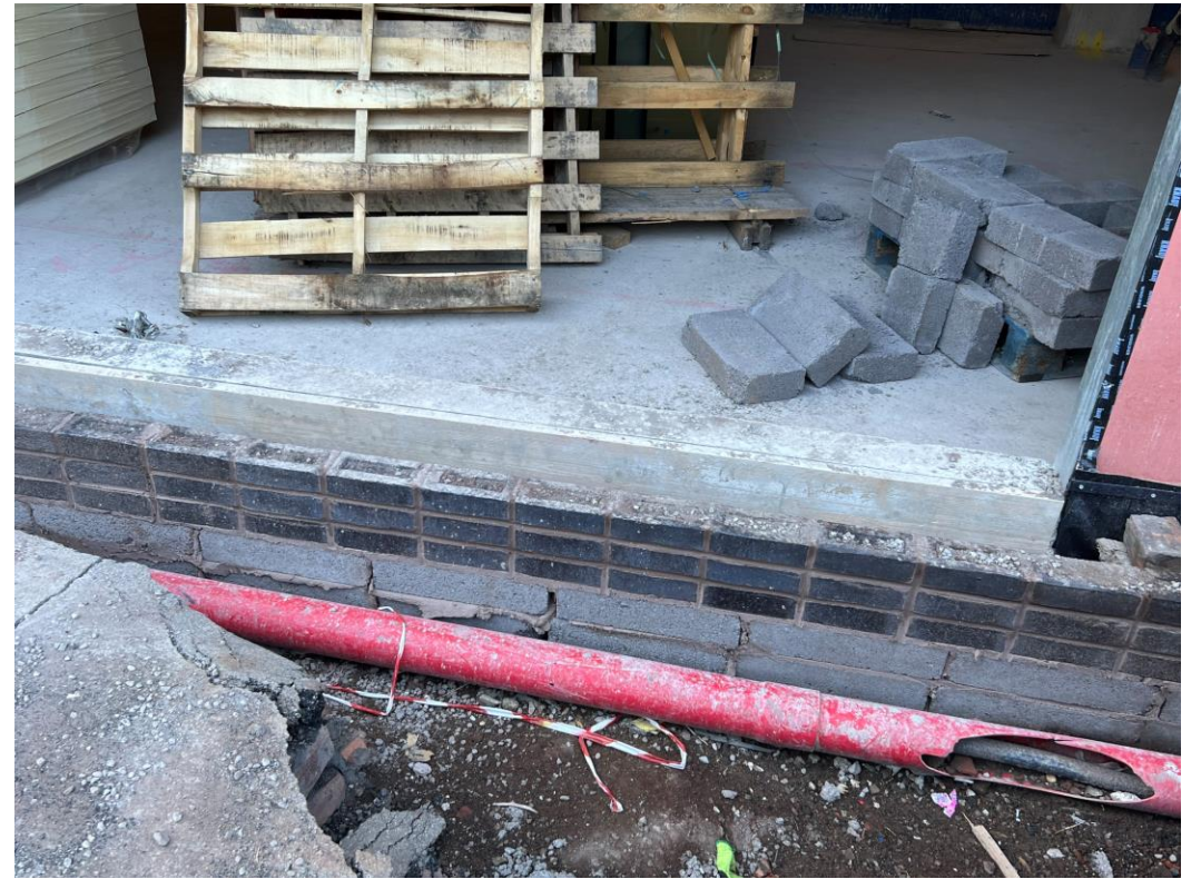
Block B Sub-structure brickwork
