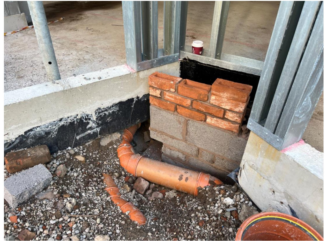
Block B Sub-structure brickwork
