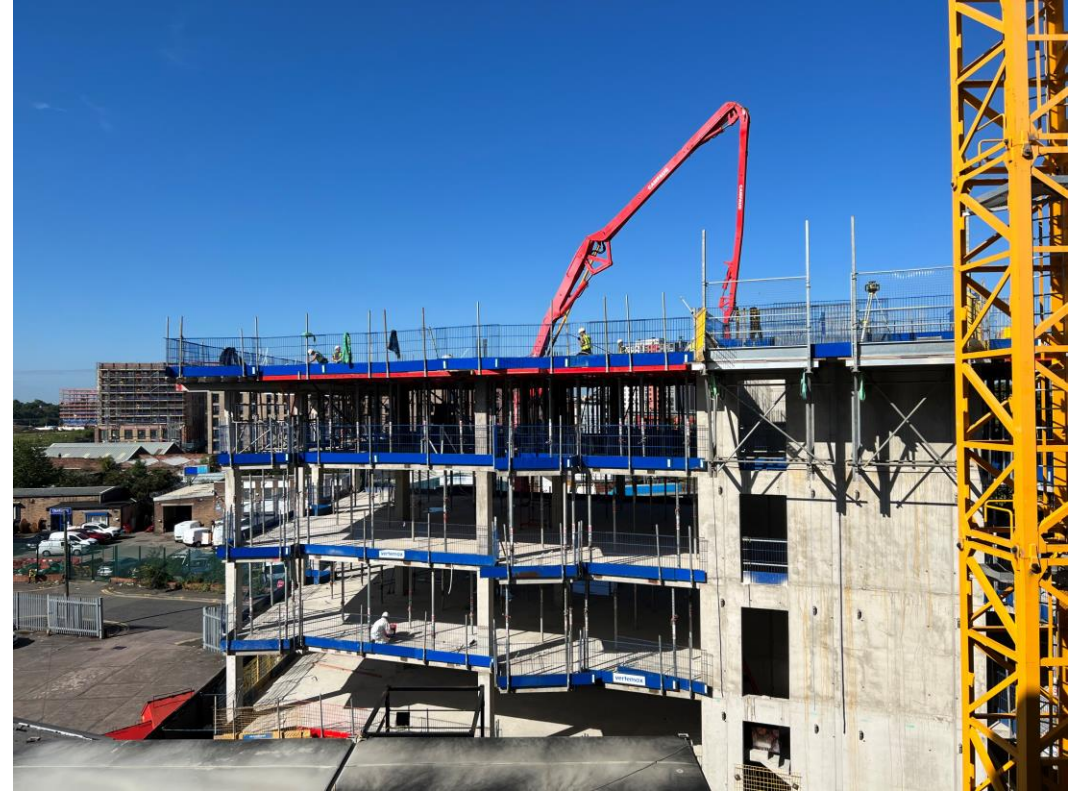
Block A concrete framework
