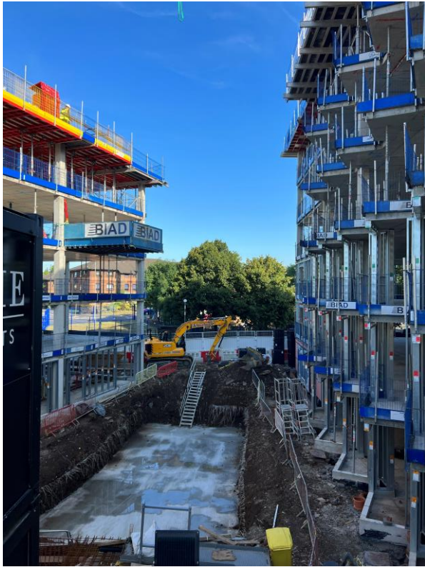
Block A & B concrete framework
