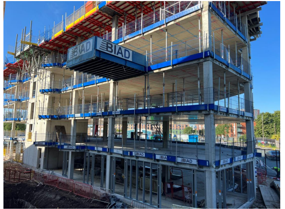
Block A concrete framework
