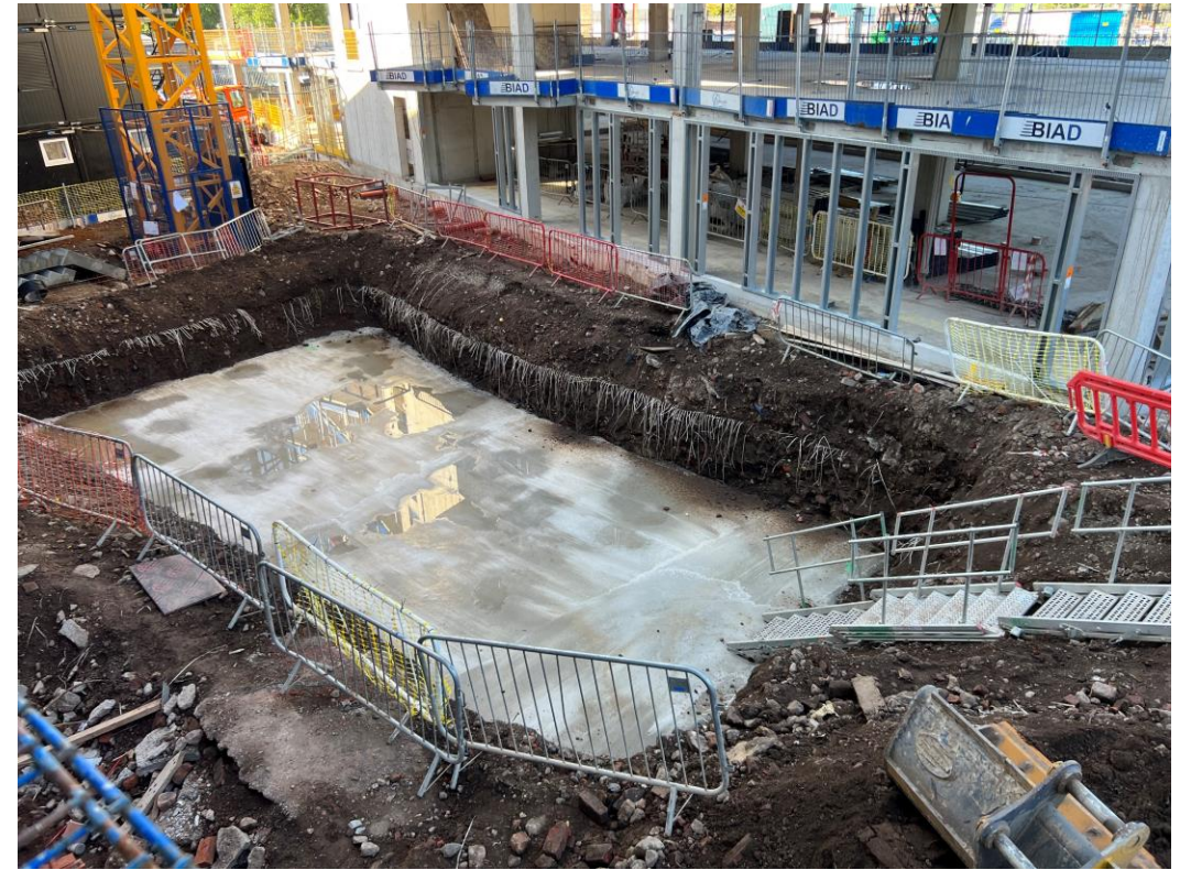
Block A & B attenuation drainage preparation
