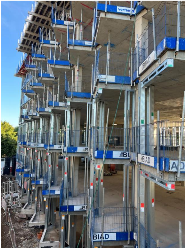
Block B concrete framework
