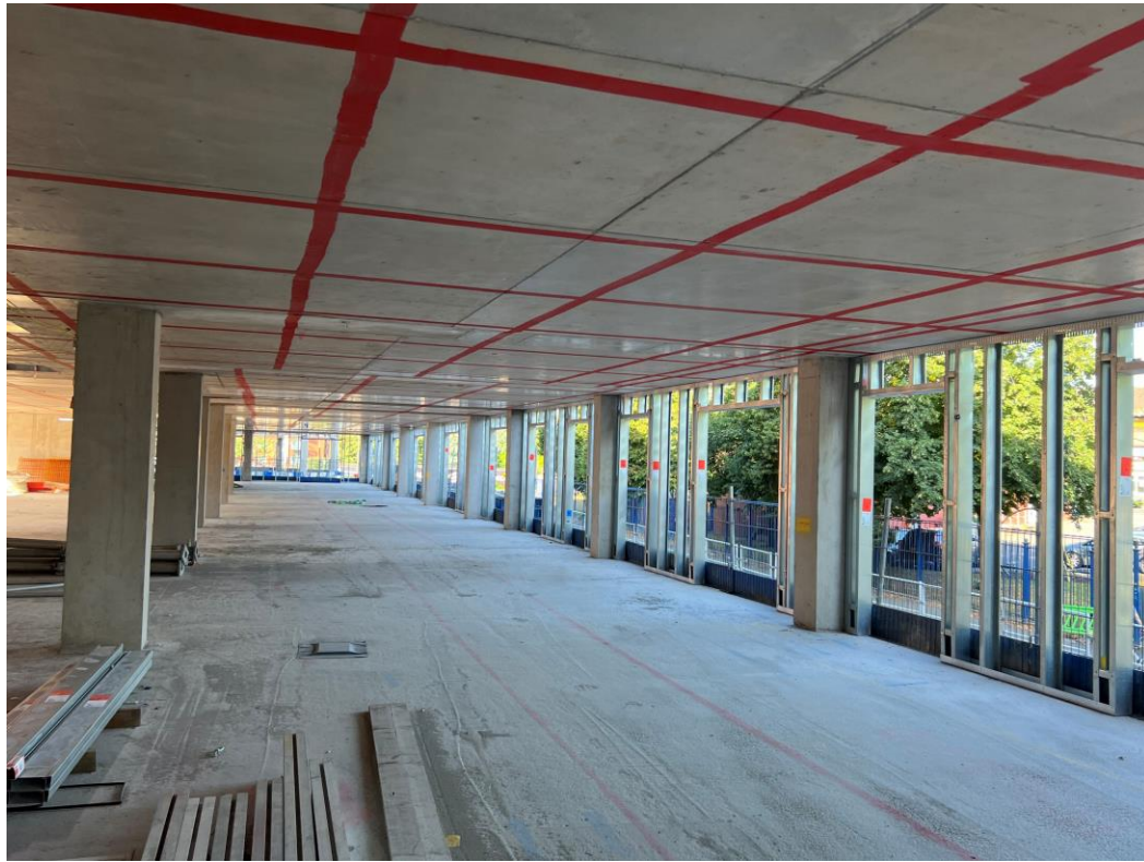
Block B First Floor concrete structure
