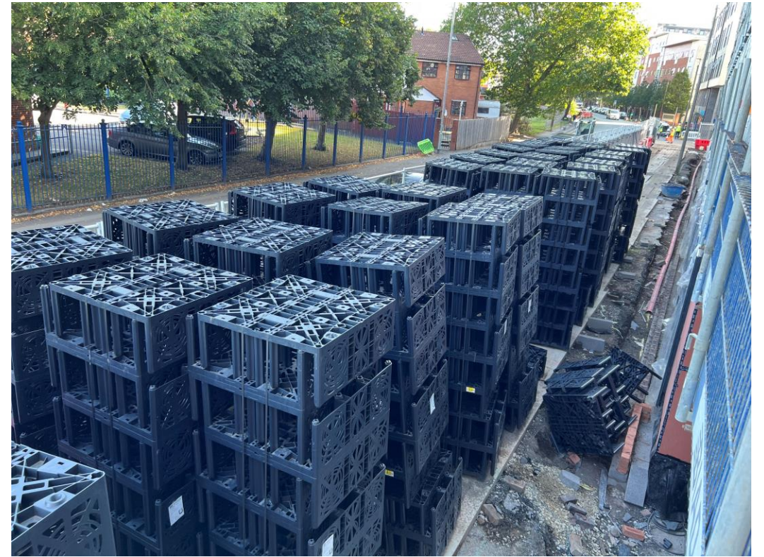
Block A & B attenuation drainage preparation
