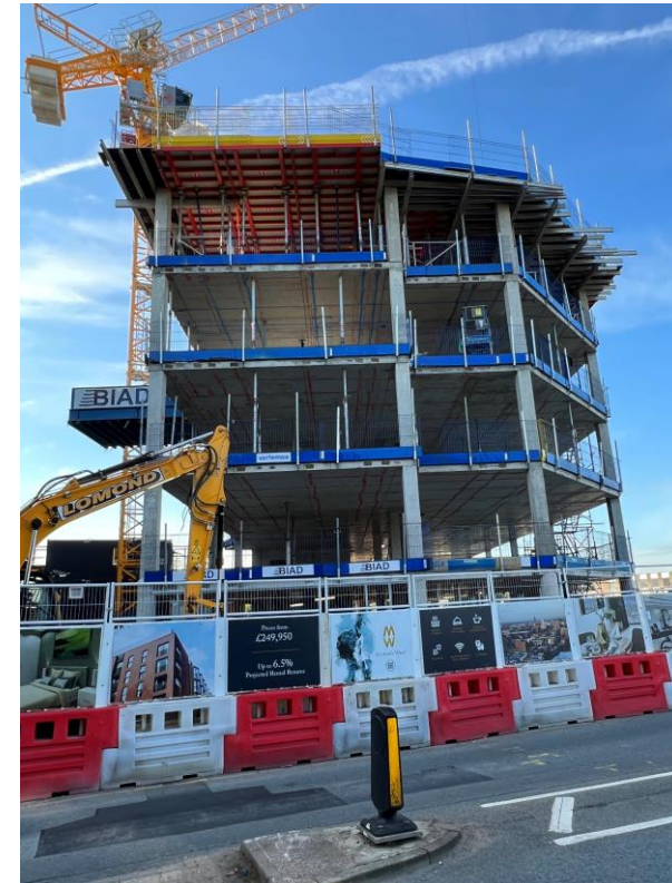
Ordsall Lane site view
