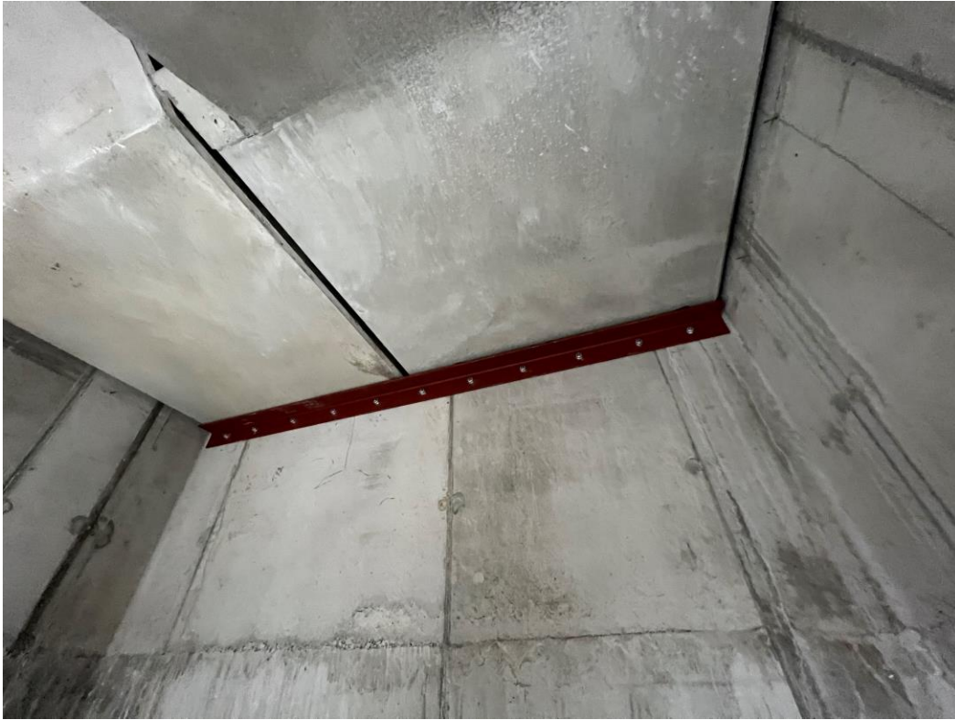
Block B concrete staircase
