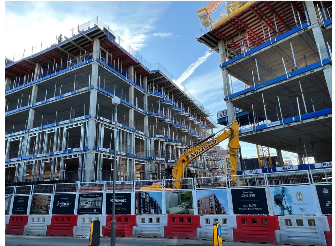
Ordsall Lane site view
