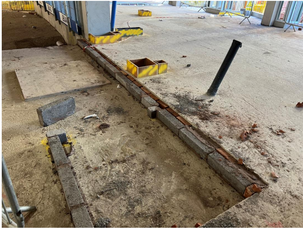
Block B ground floor internal block wall
