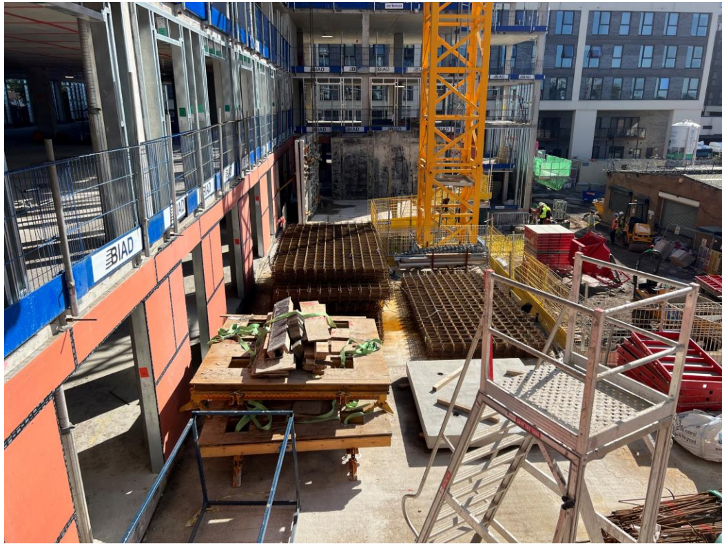
Block B structure and weatherboarding
