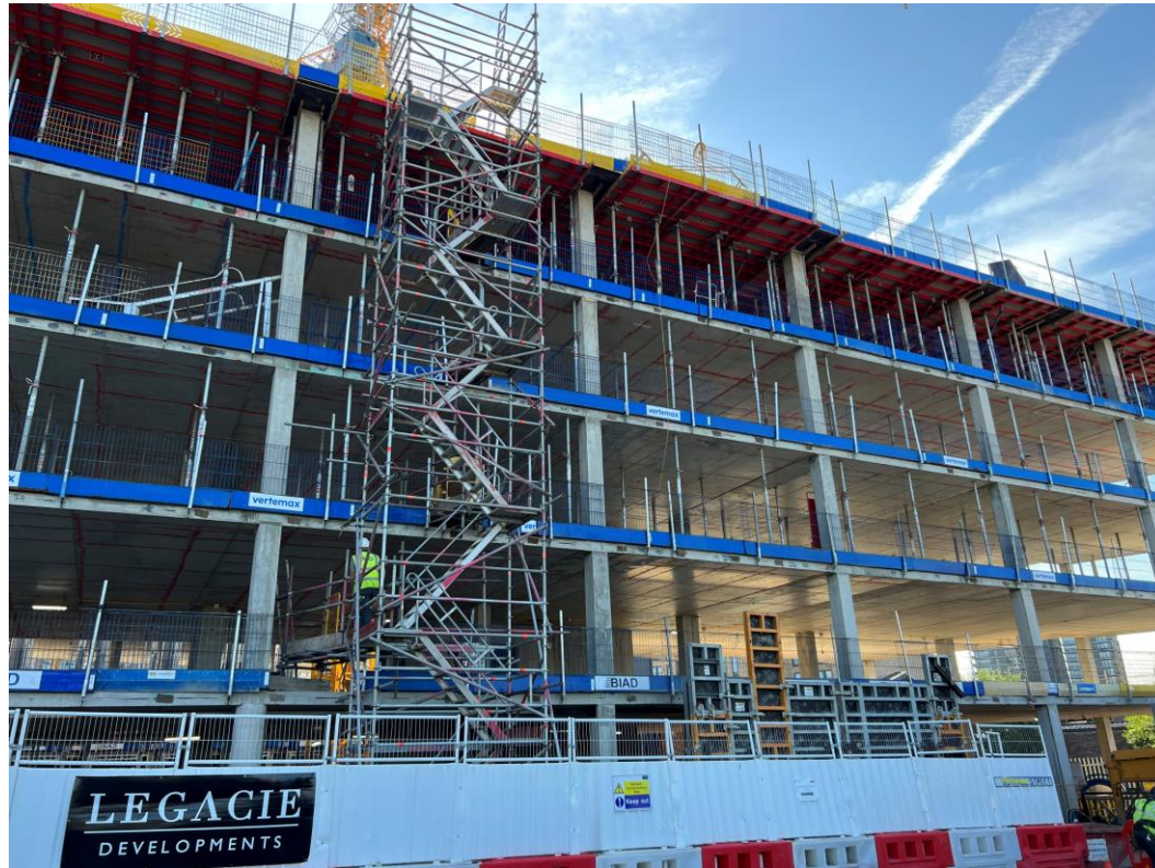
Ordsall Lane site view
