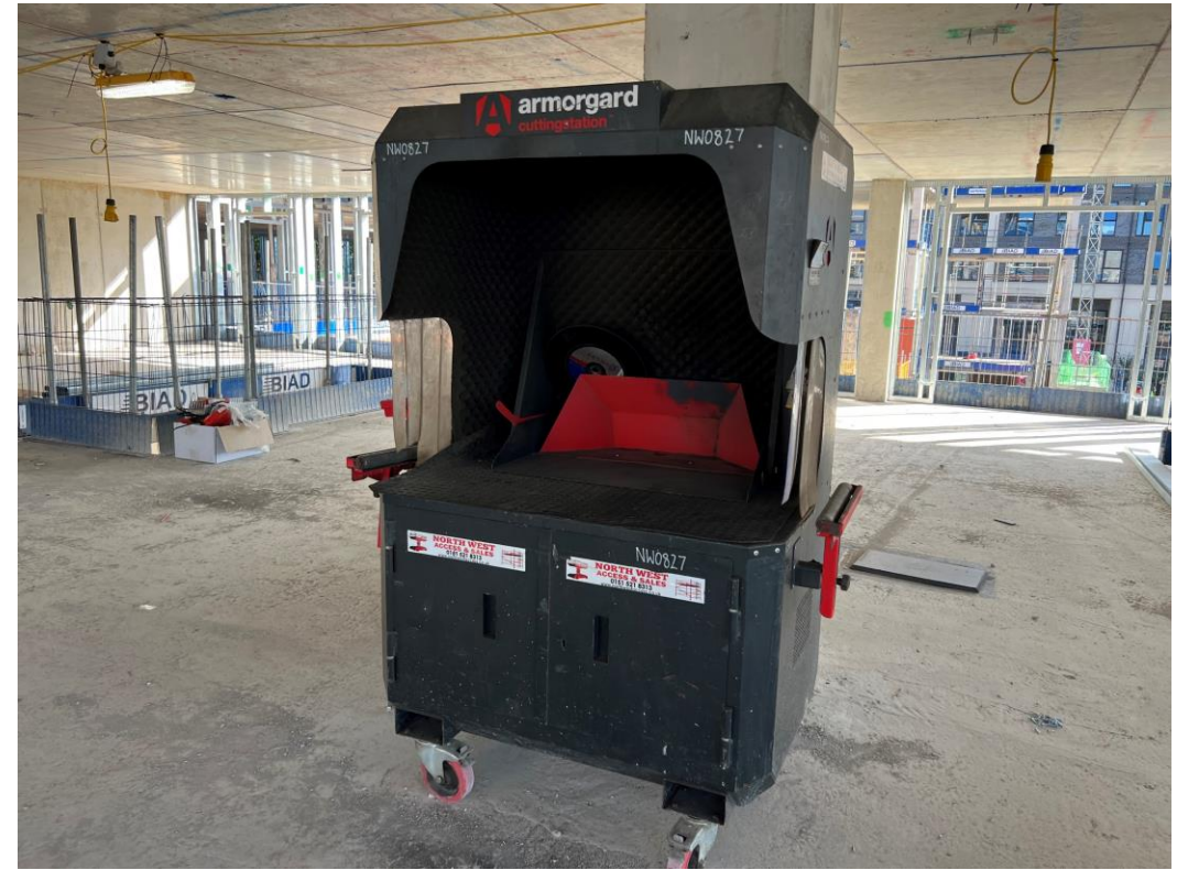
Block B Second Floor SFS structure
