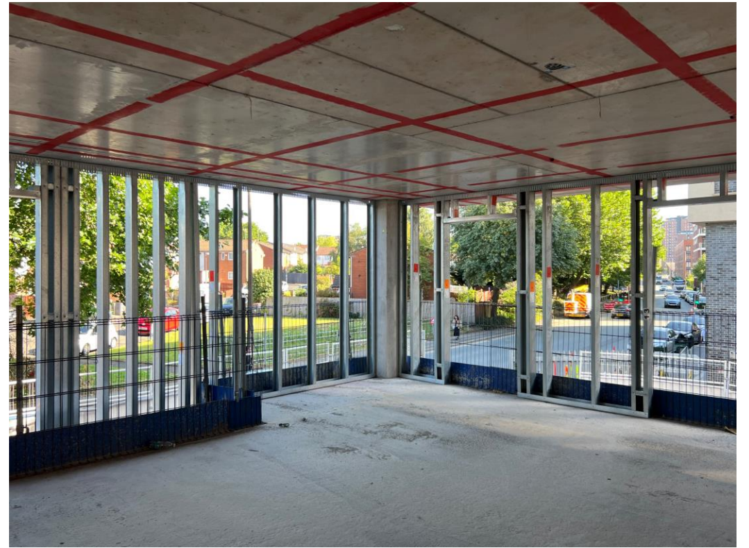
Block B First Floor SFS
