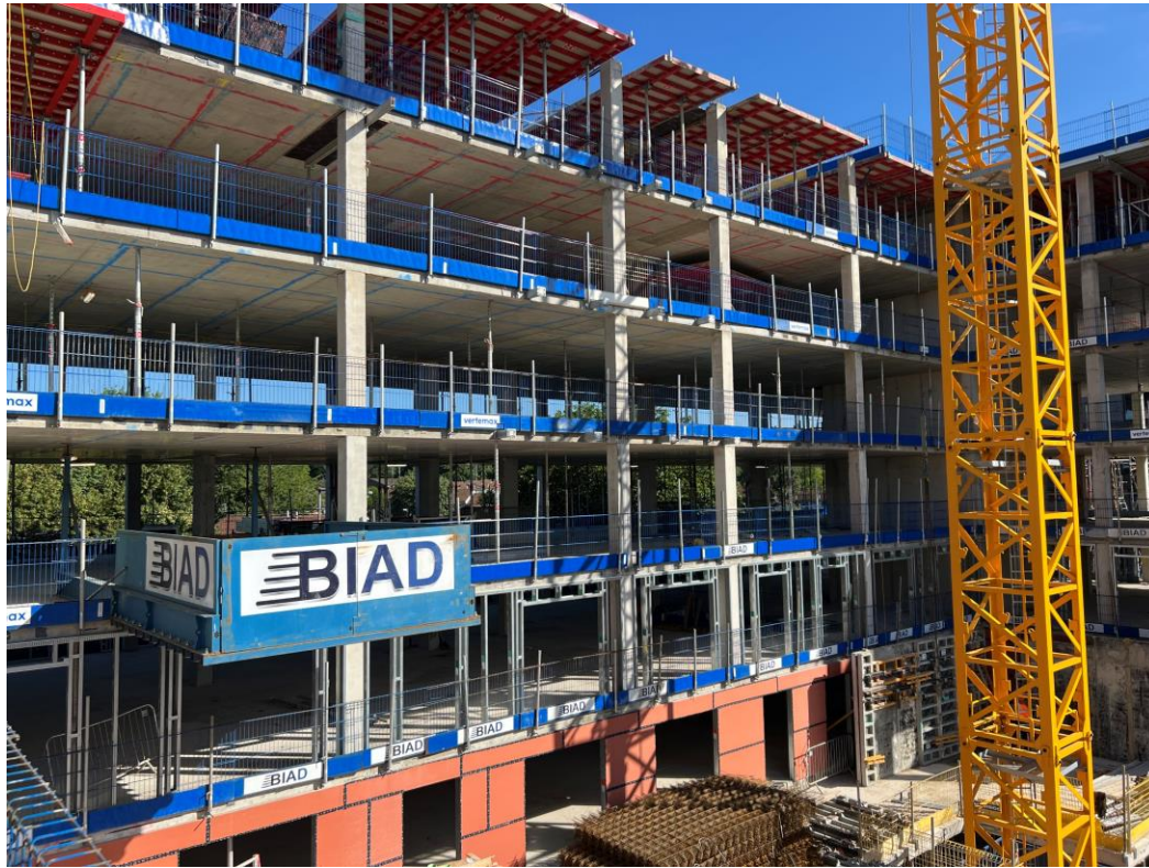
Block B structure and weatherboarding
