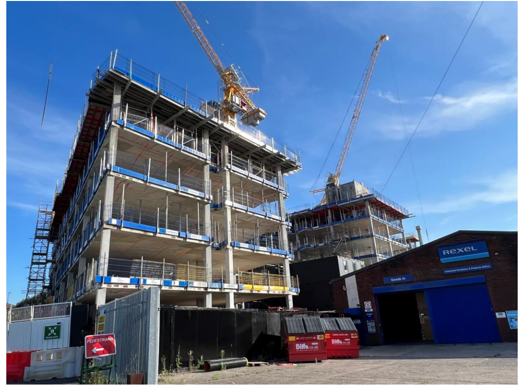
Worrall Street site view
