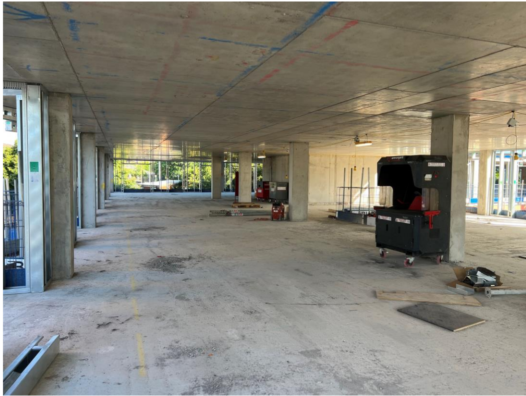
Block B Second Floor concrete structure
