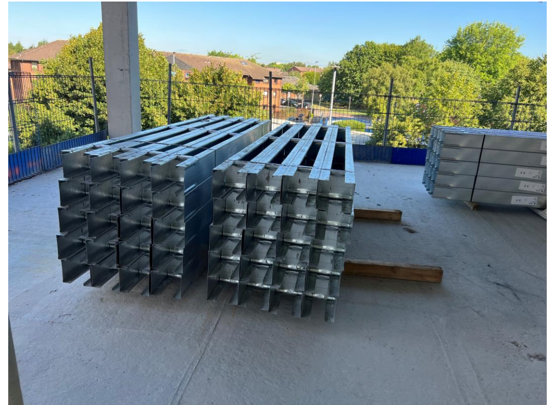
Block B Third Floor SFS materials
