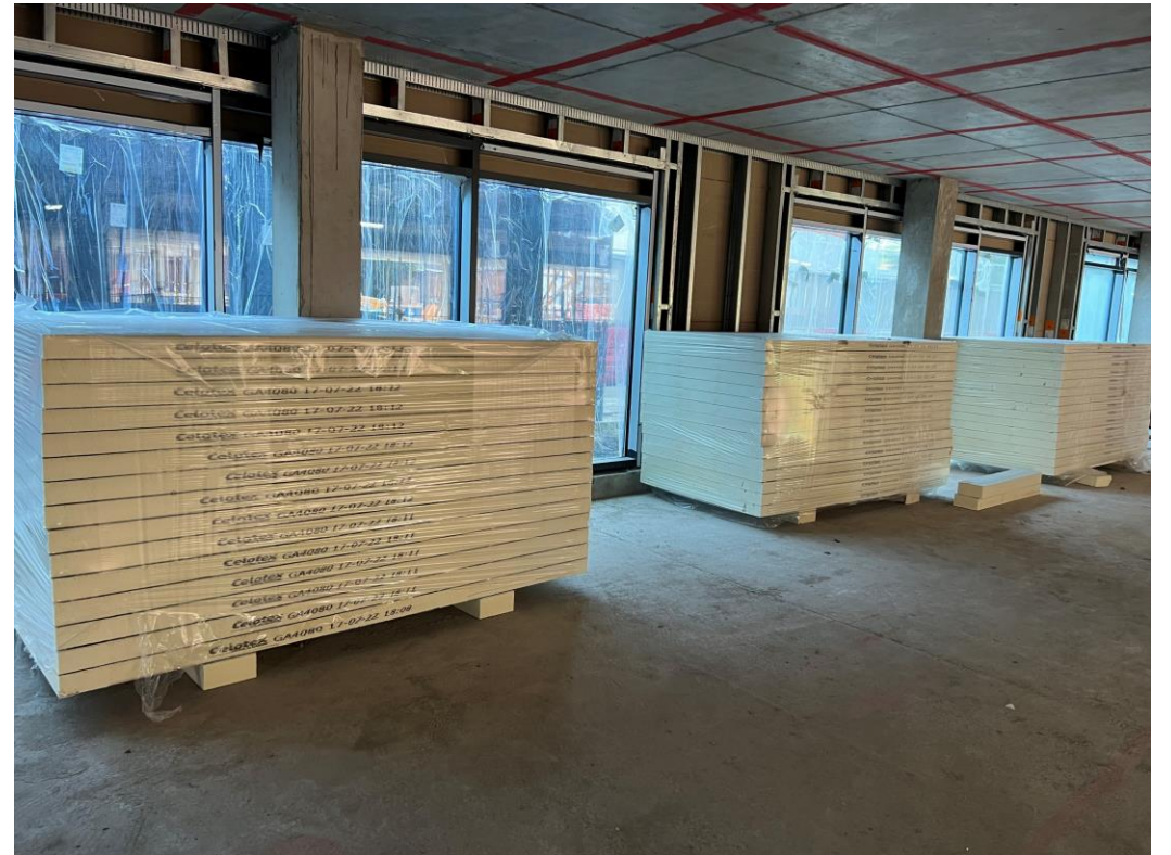
Block B wall insulation stored
