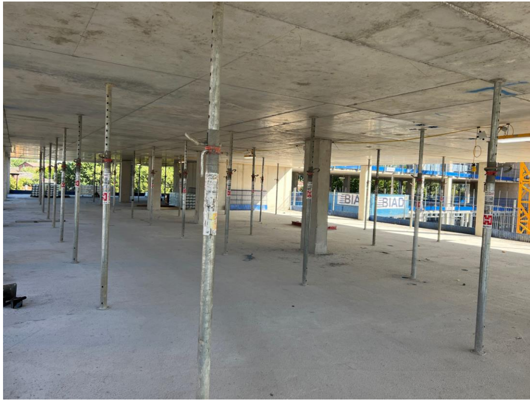
Block B Third Floor concrete structure
