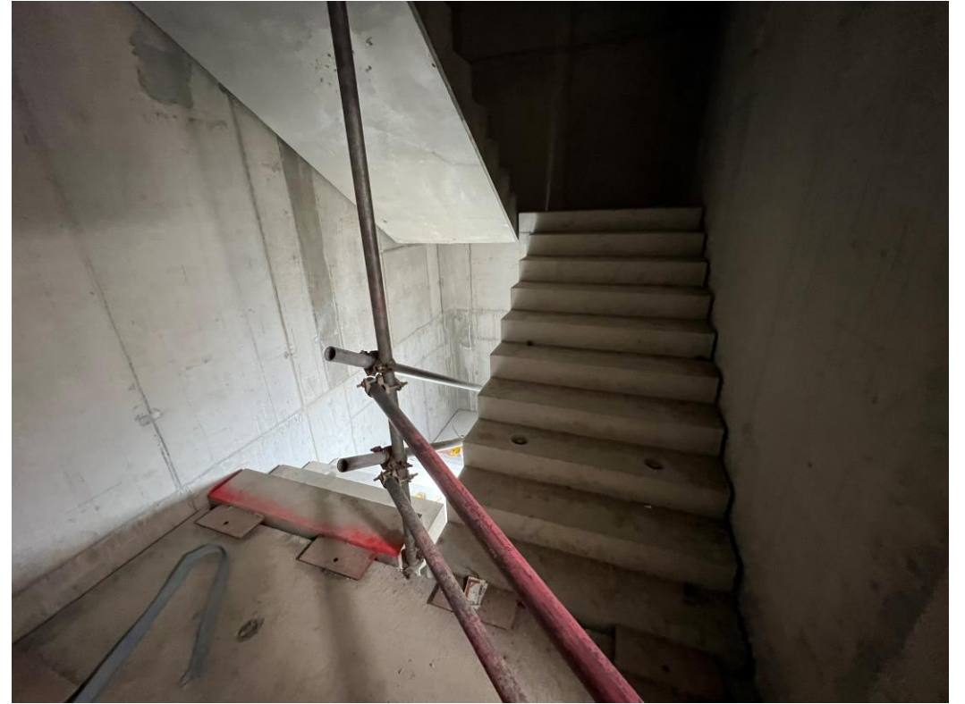
Block B concrete staircase
