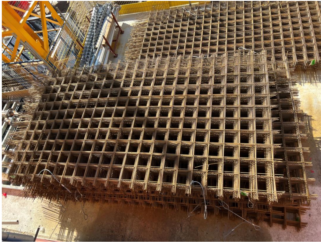
Block B reinforcement stored
