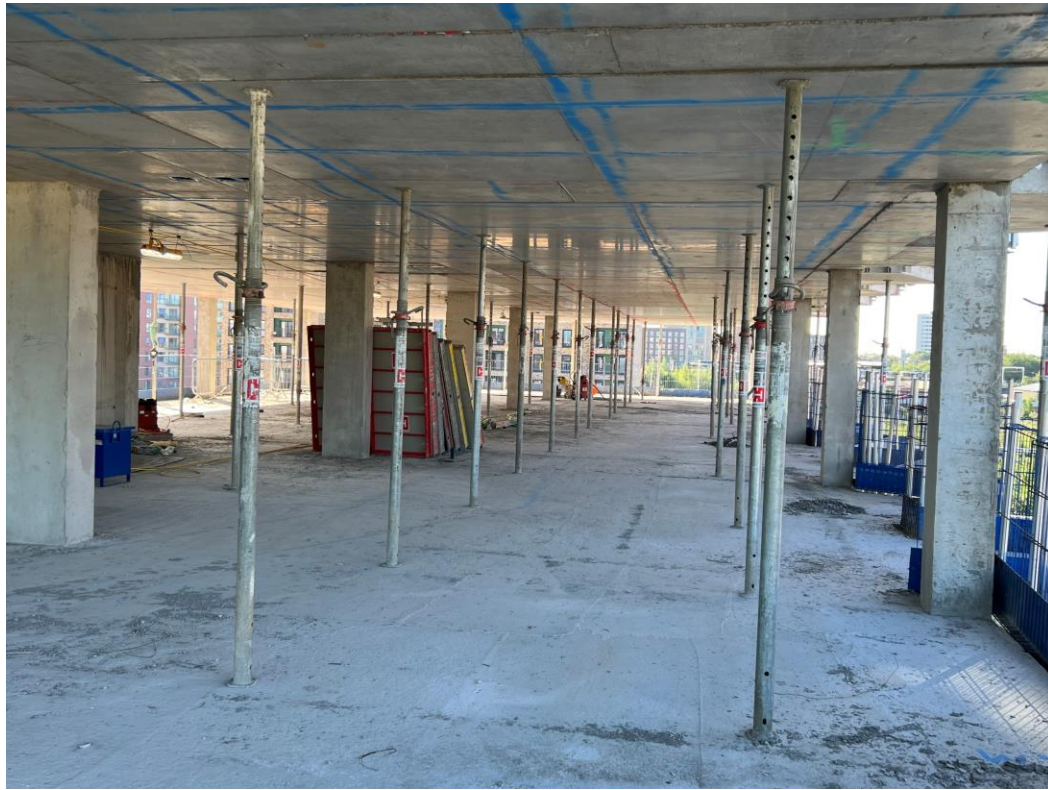
Block B Fourth Floor concrete structure
