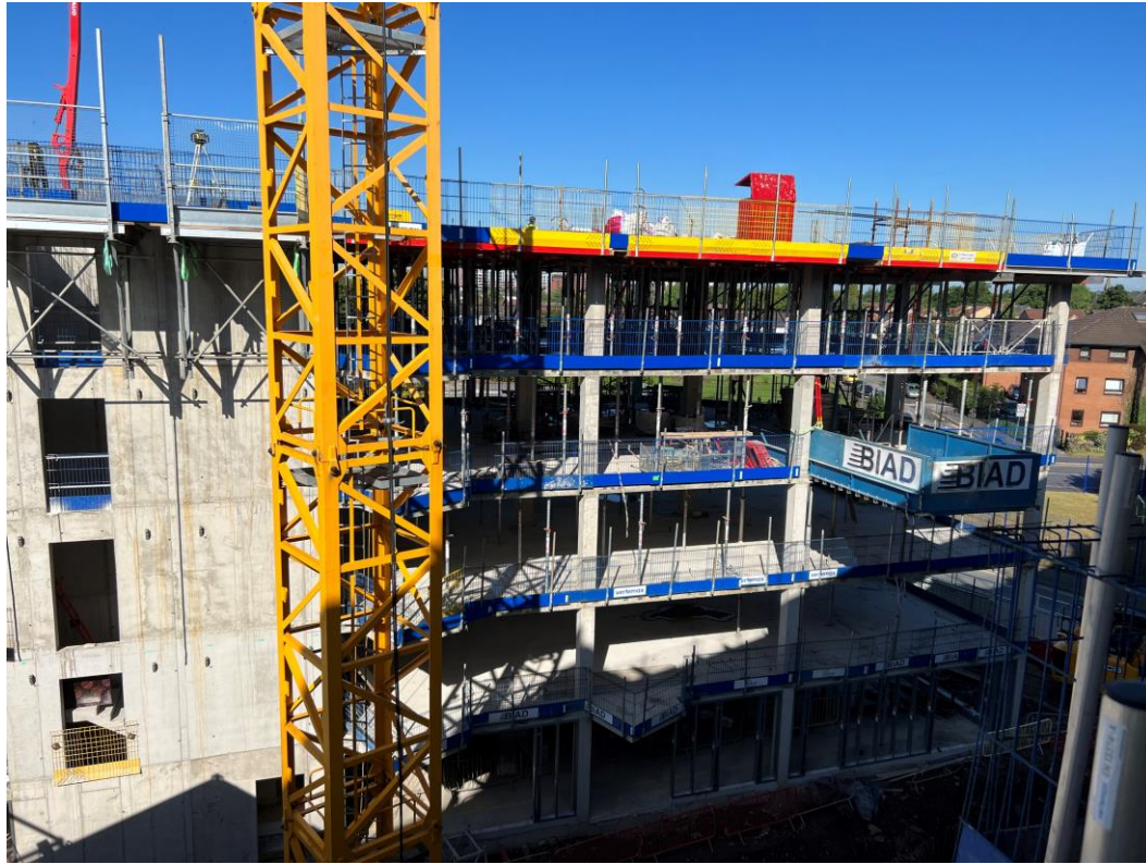
Block A concrete framework
