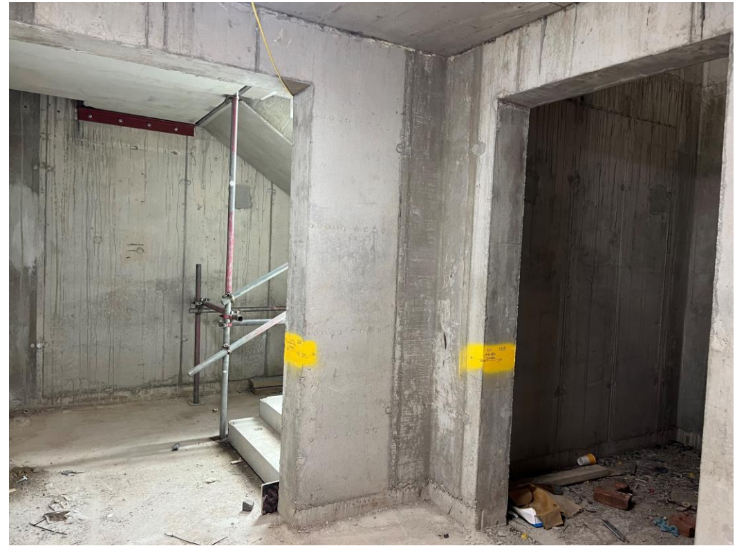
Block B stair and lift core
