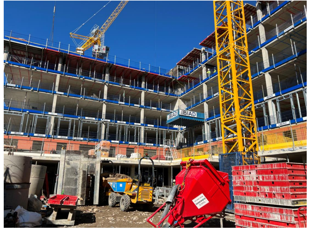
Block B weatherboarding
