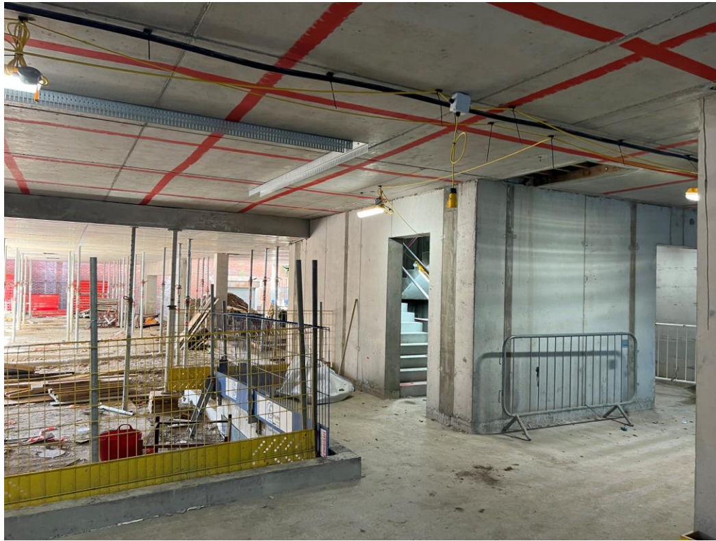
Block B stair core
