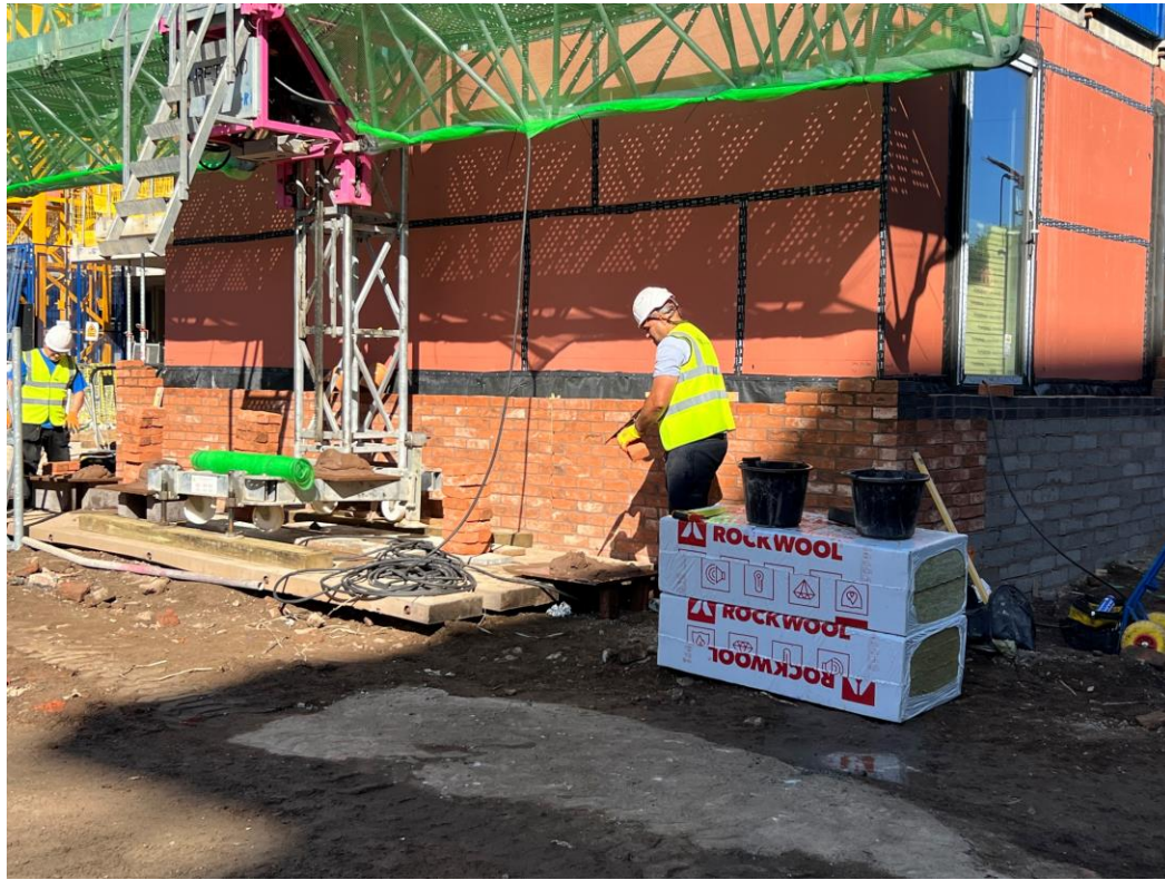
Block B Facing brickwork
