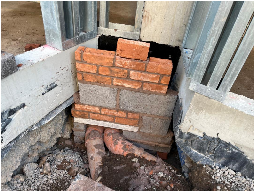
Block B Sub-structure brickwork
