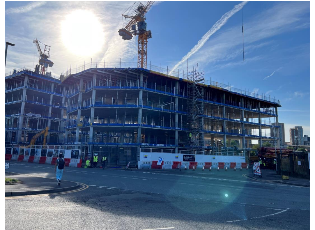
Ordsall Lane site view
