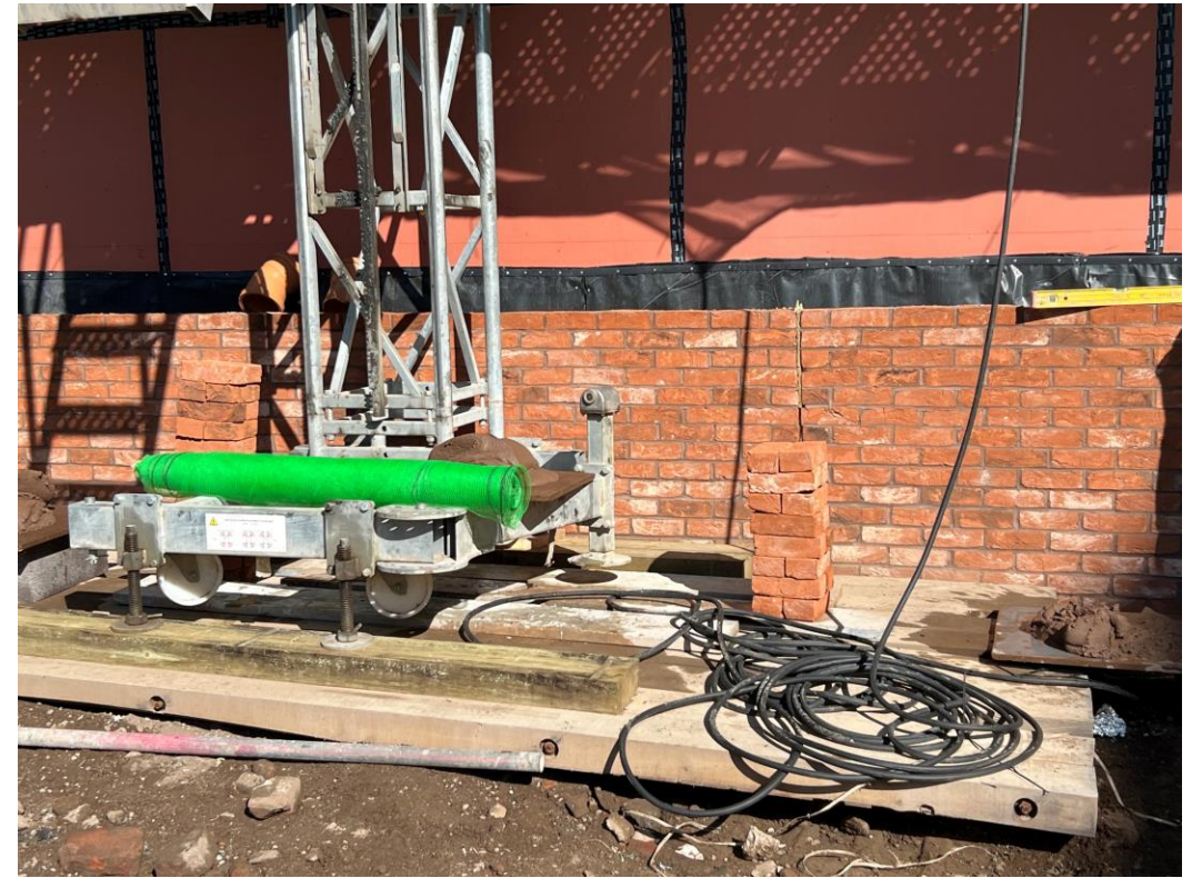
Block B Facing brickwork
