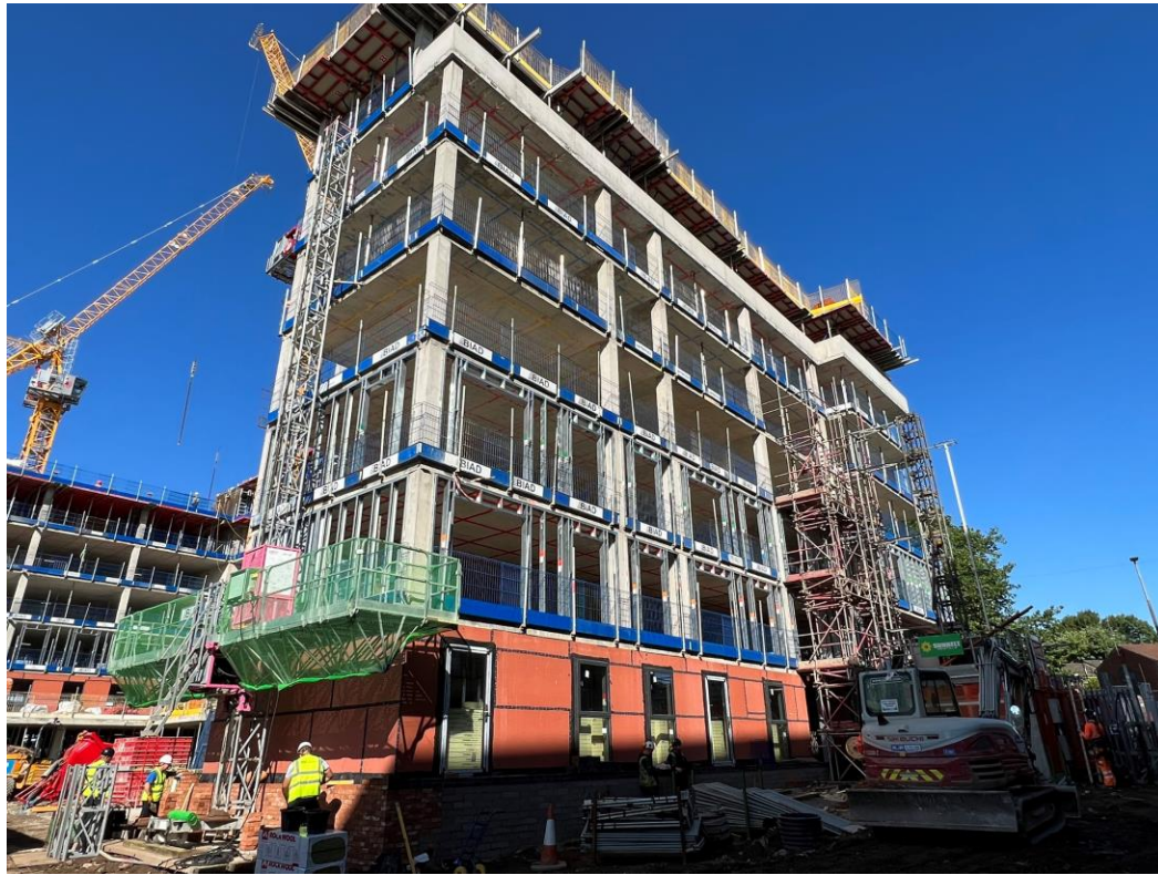
Block B mast climber & hoist access installed
