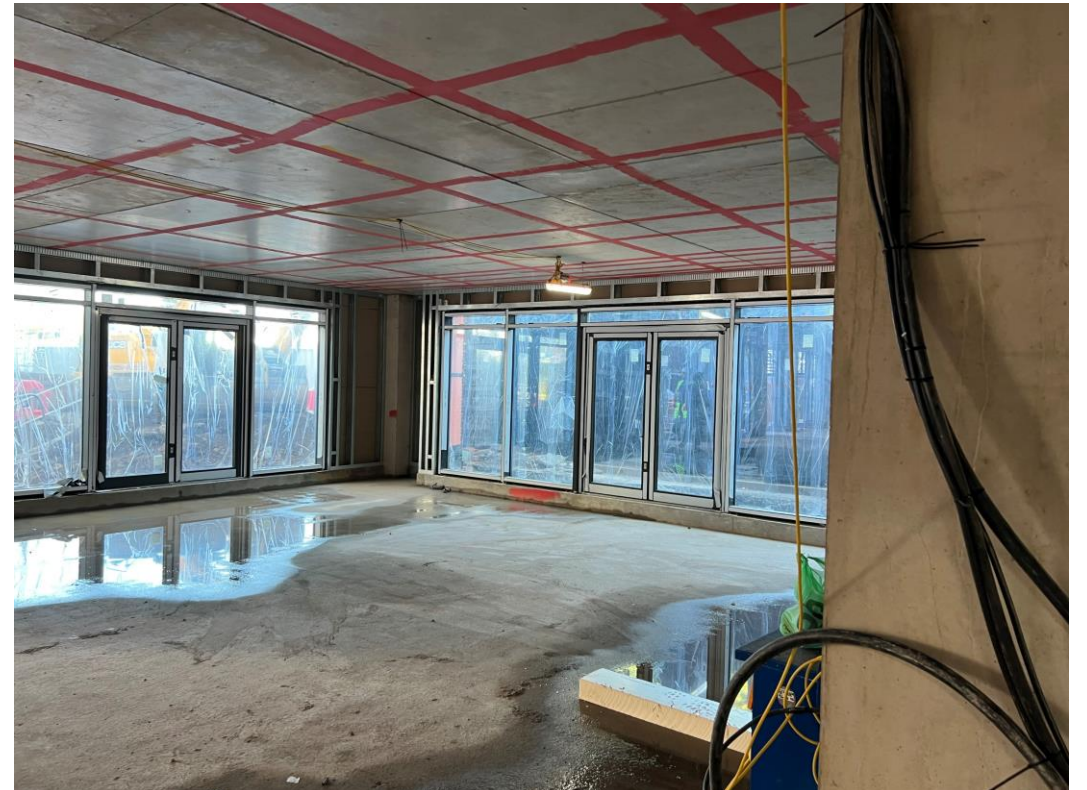
Block B windows and doors
