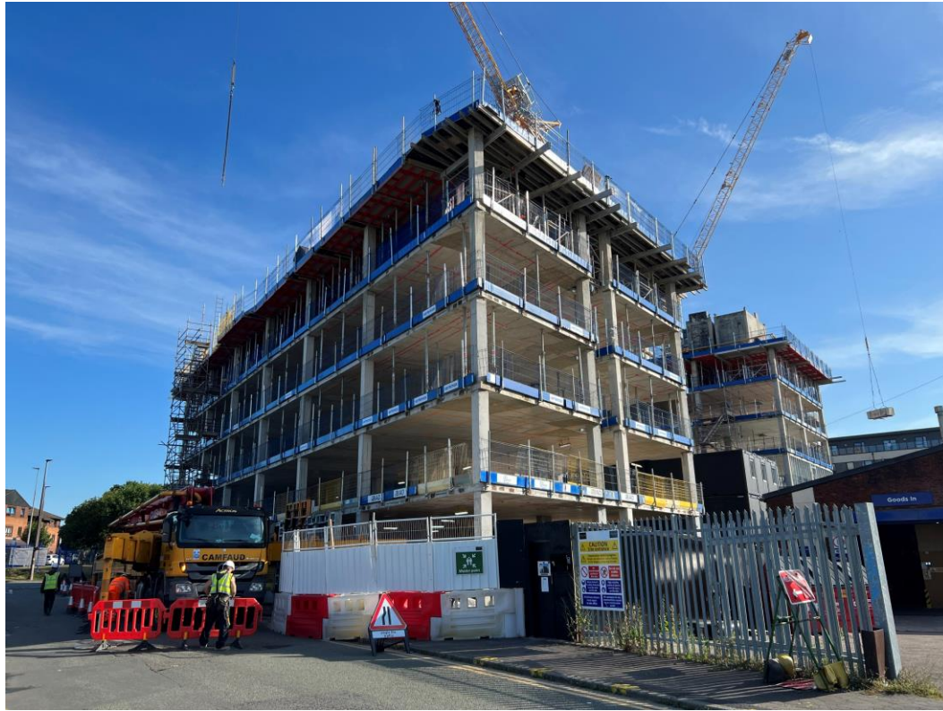
Worrall Street site view
