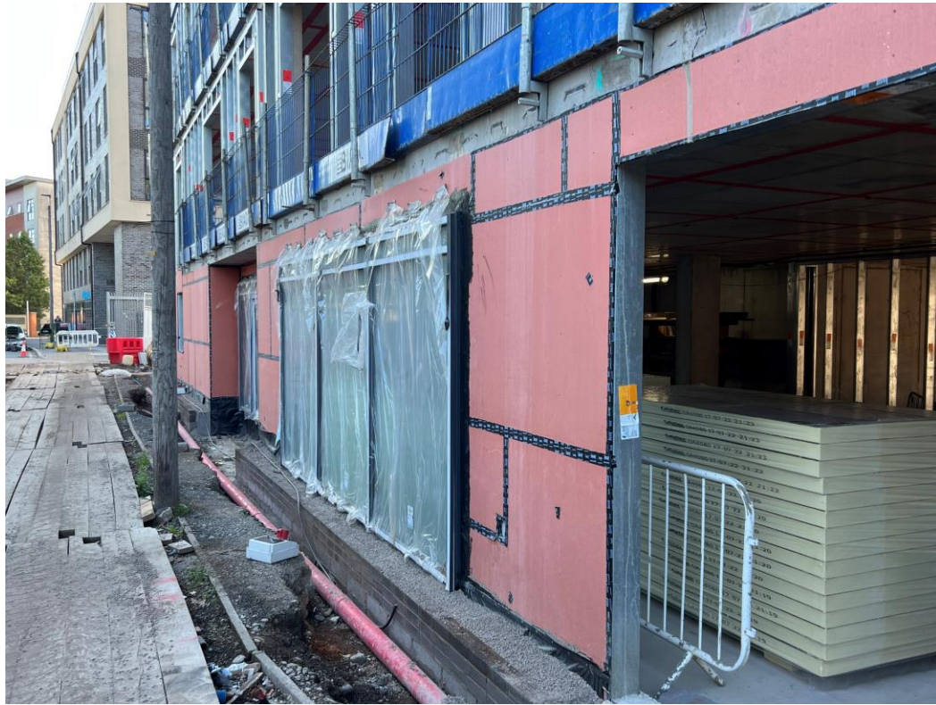
Block B Sub-structure brickwork
