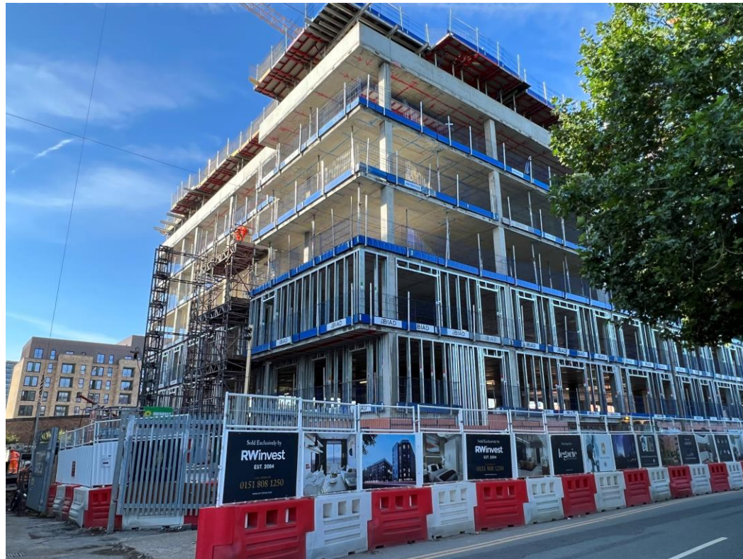
Ordsall Lane site view
