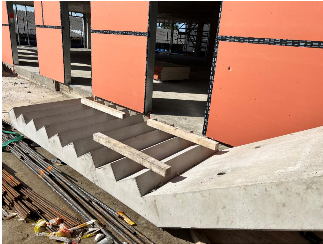
Block B staircase stored
