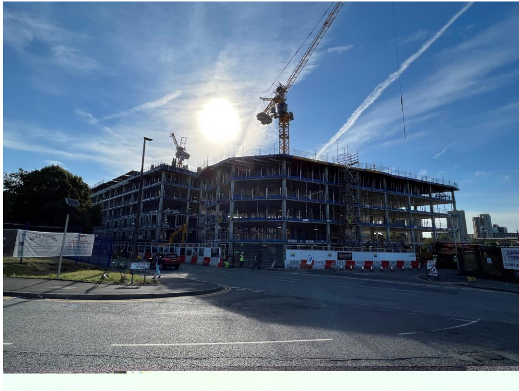
Ordsall Lane site view
