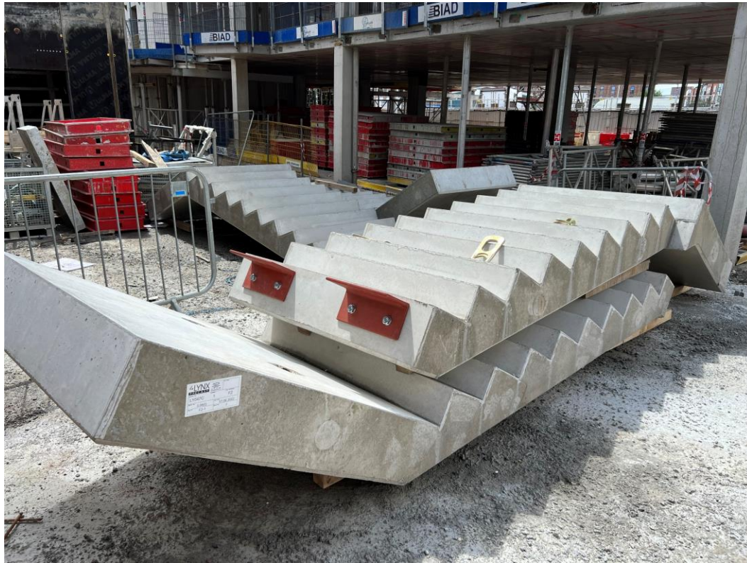
Block B concrete staircase stored
