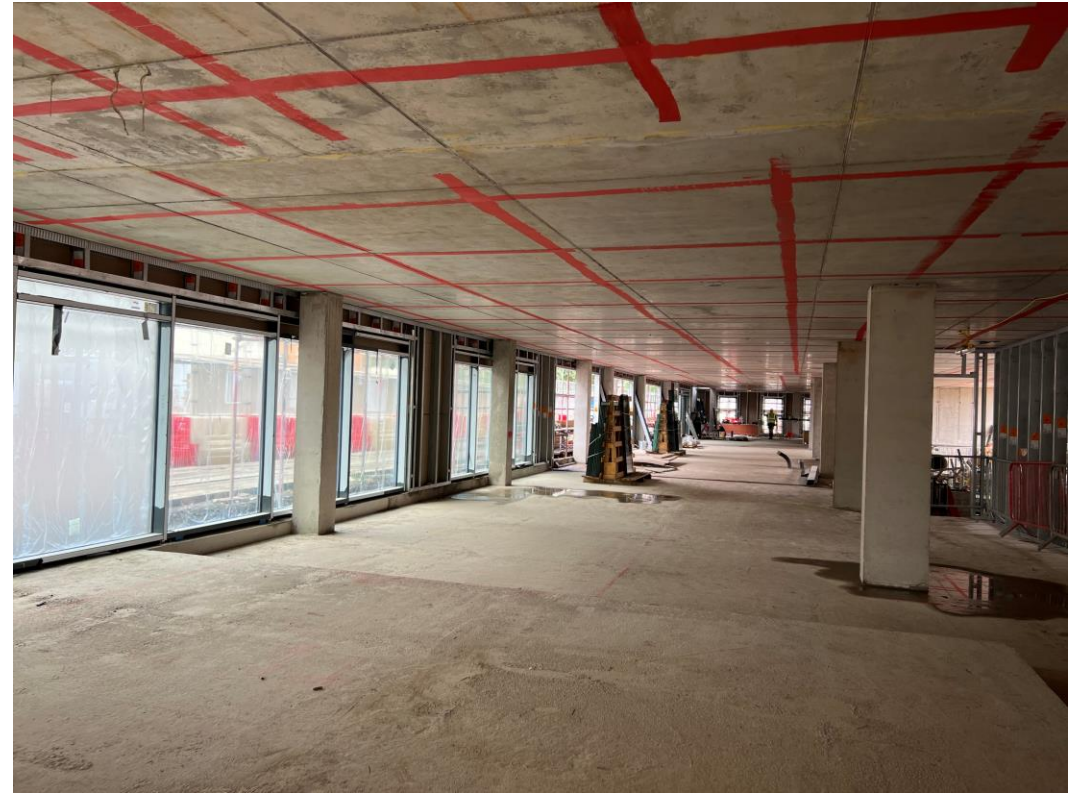
Block B ground floor windows installed
