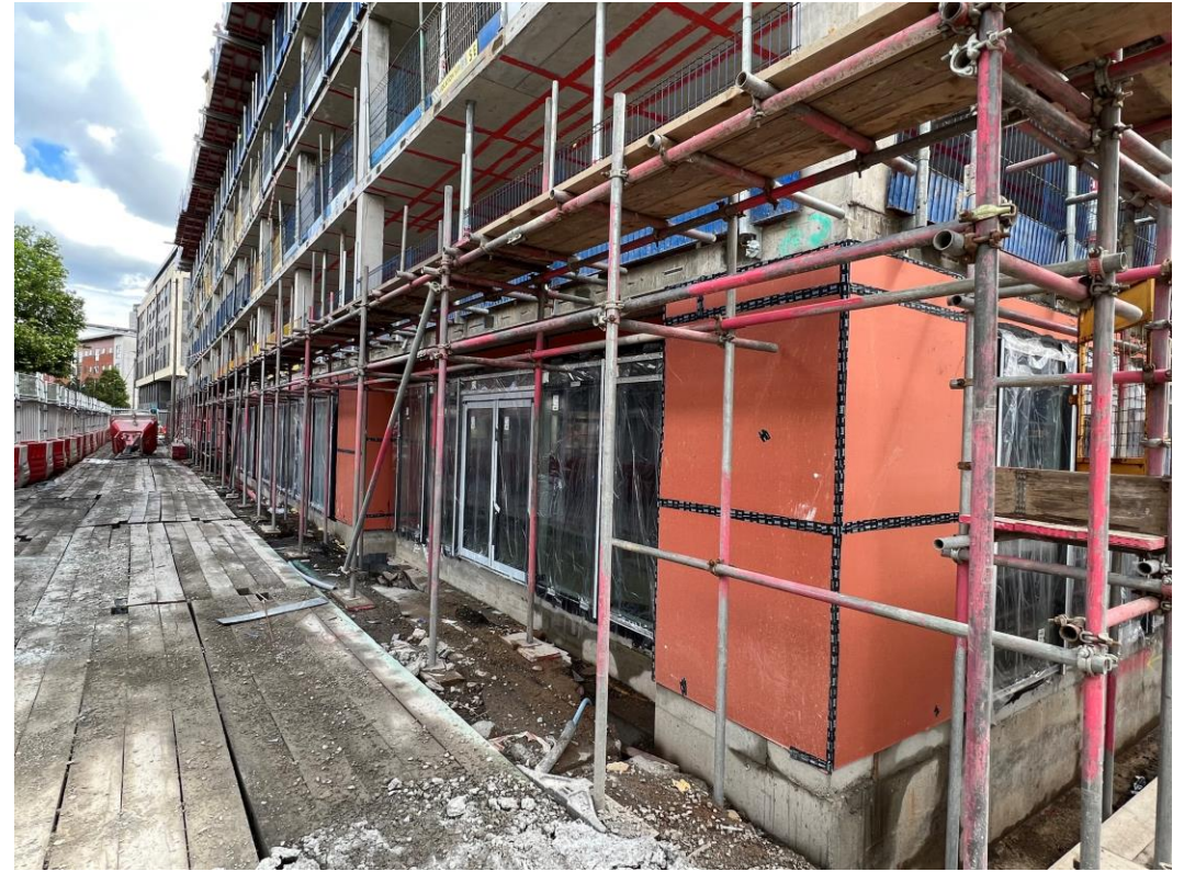
Block B external windows & doors
