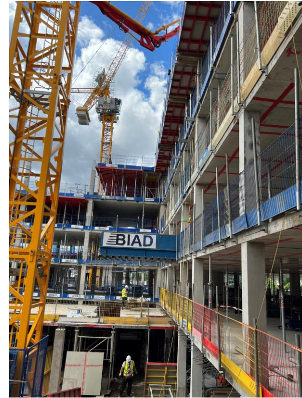
Block B concrete framework
