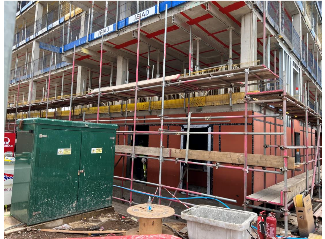
Block B SFS & weatherboarding
