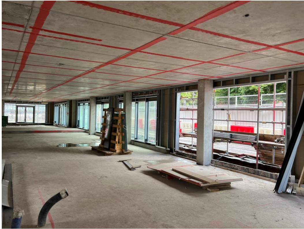
Block B ground floor windows installed
