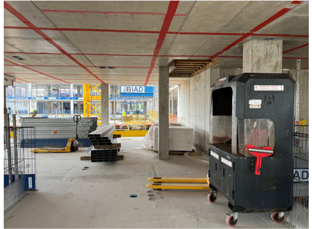
Block B first floor SFS cutter
