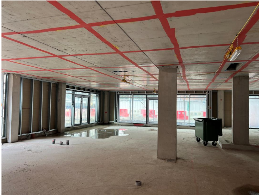
Block B ground floor windows installed
