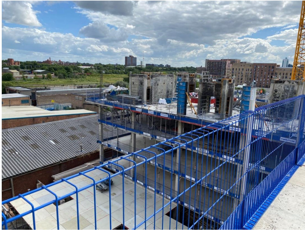
Block B concrete frame under construction
