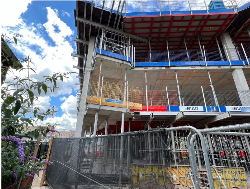
Block A concrete framework
