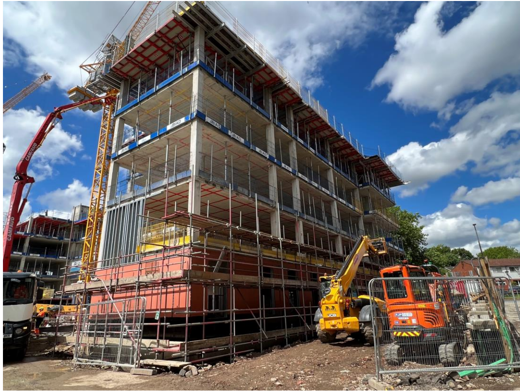
Block B SFS & weatherboarding
