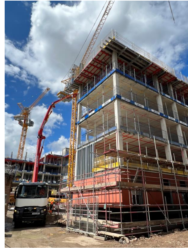
Block B SFS framework & weatherboarding
