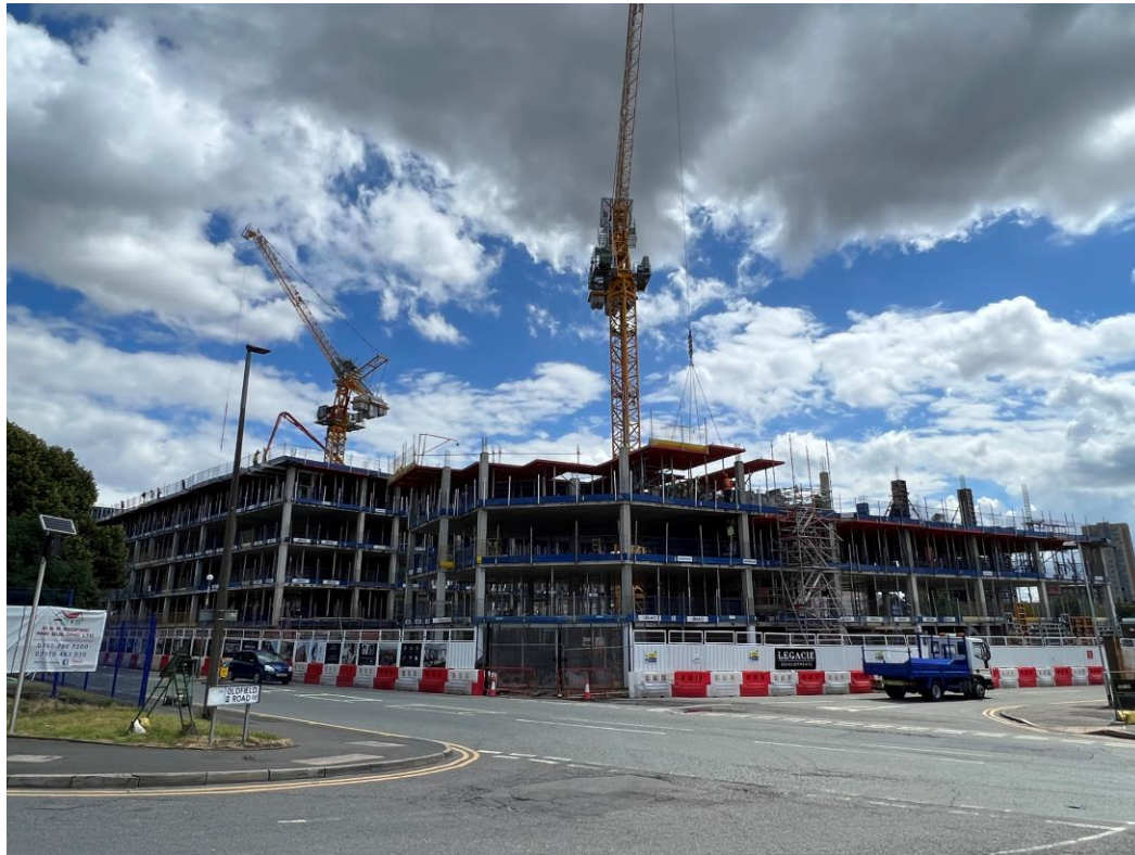
Ordsall Lane site view
