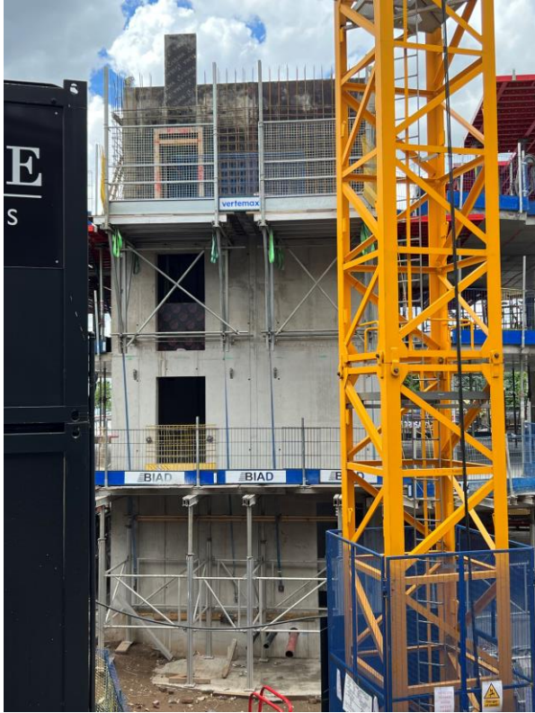
Block B stair and lift core
