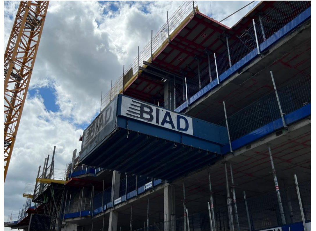
Block A hoist access
