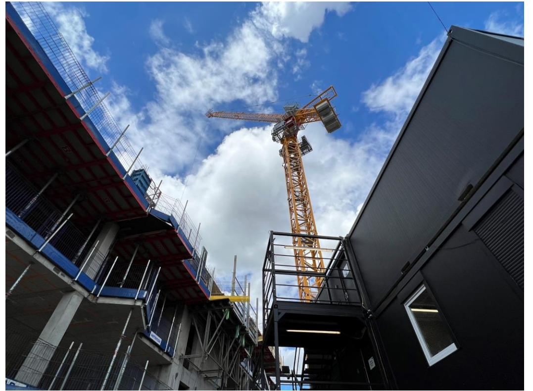
Site entrance Worrall Street
