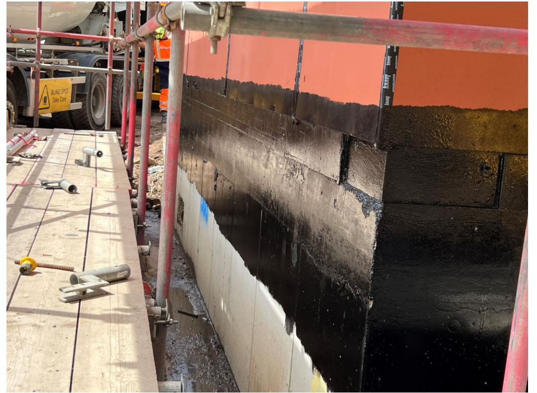
Block B SFS & weatherboarding & tanking
