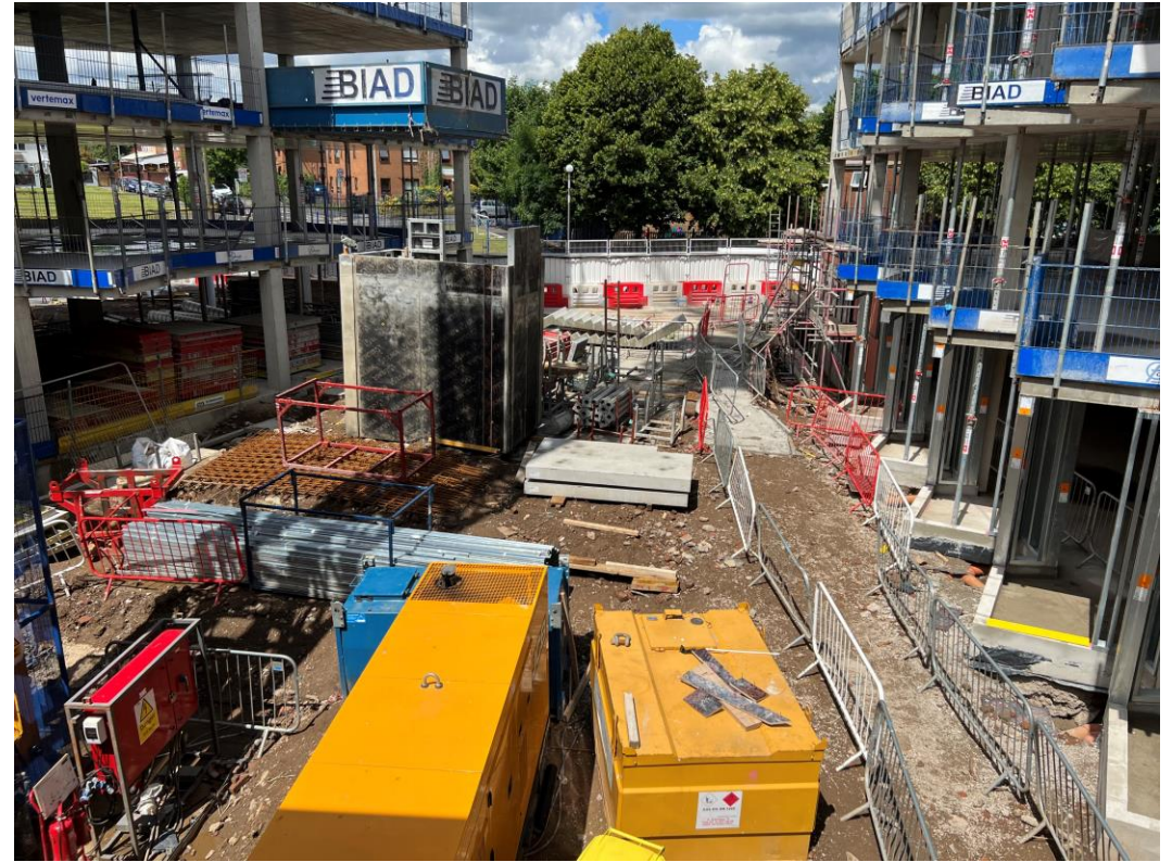
Block A & B concrete framework
