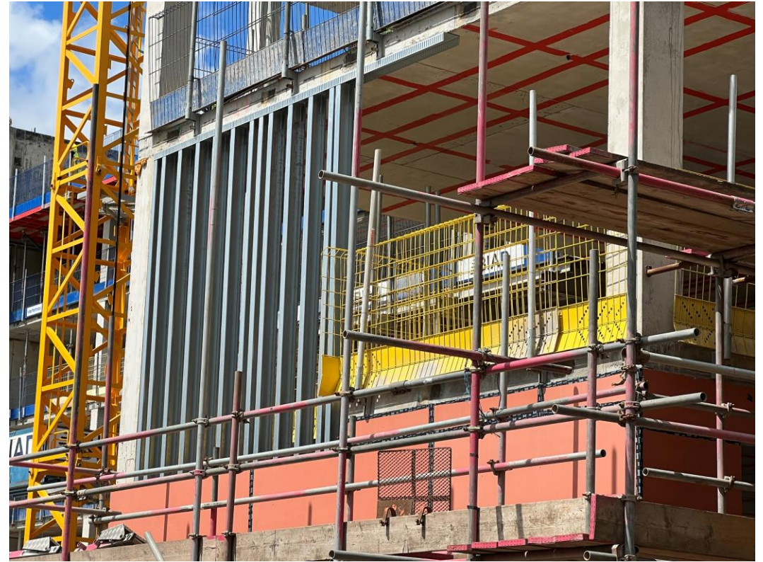
Block B SFS & weatherboarding
