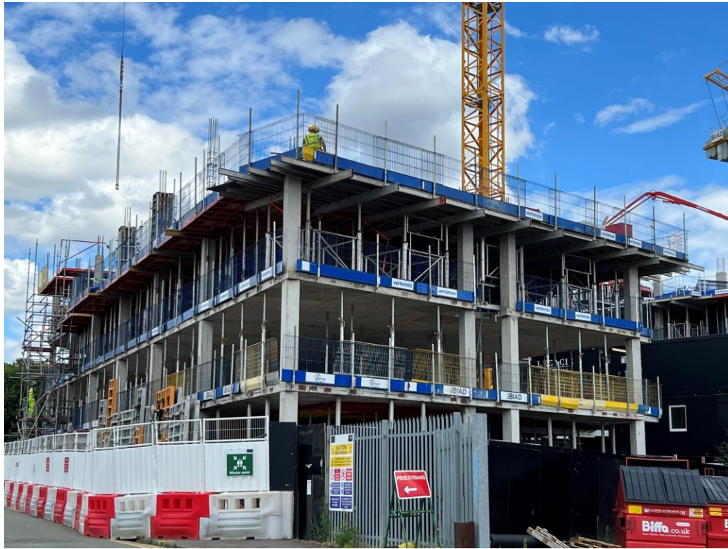
Worrall Street site view
