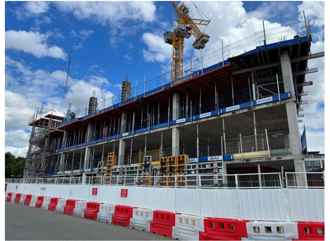
Worrall Street site view
