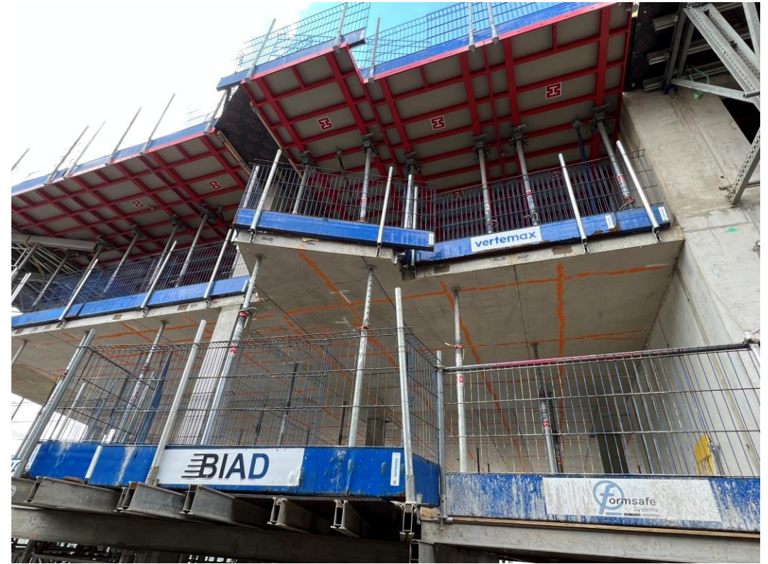
Block A concrete framework
