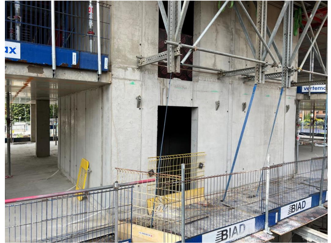
Block A stair and lift core
