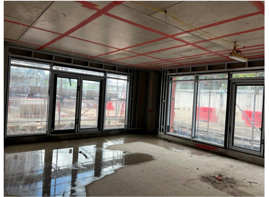
Block B ground floor windows installed
