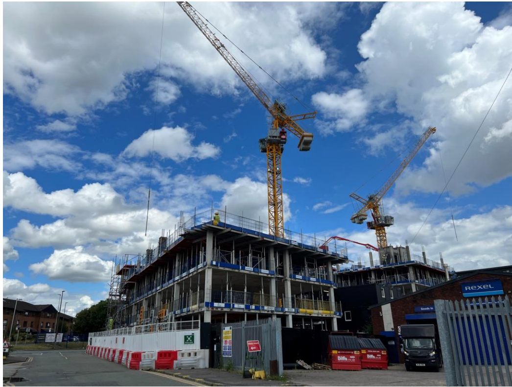
Worrall Street site view
