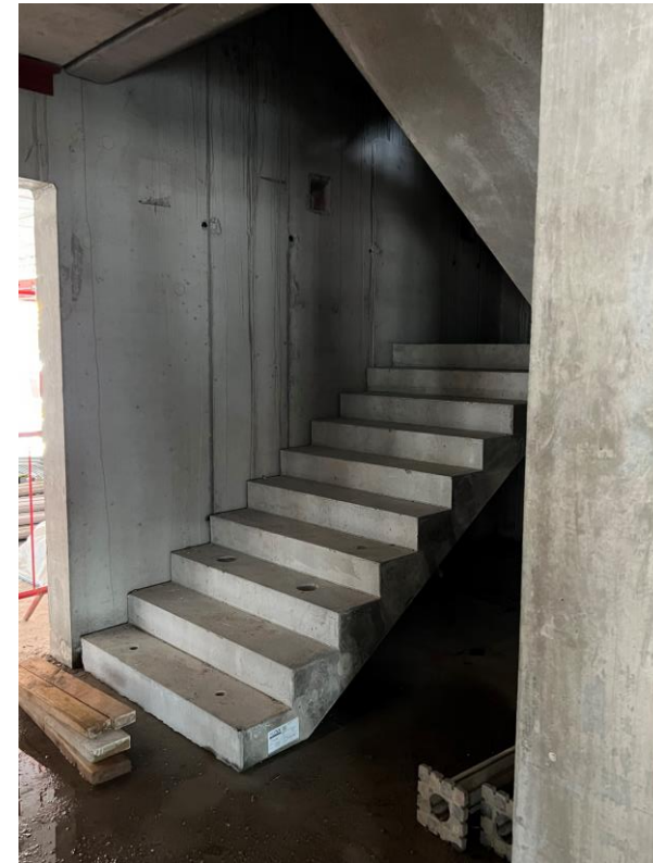
Block B staircase installed
