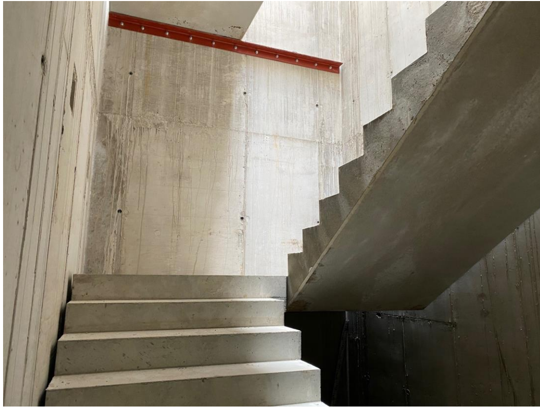
Block B concrete staircase installed
