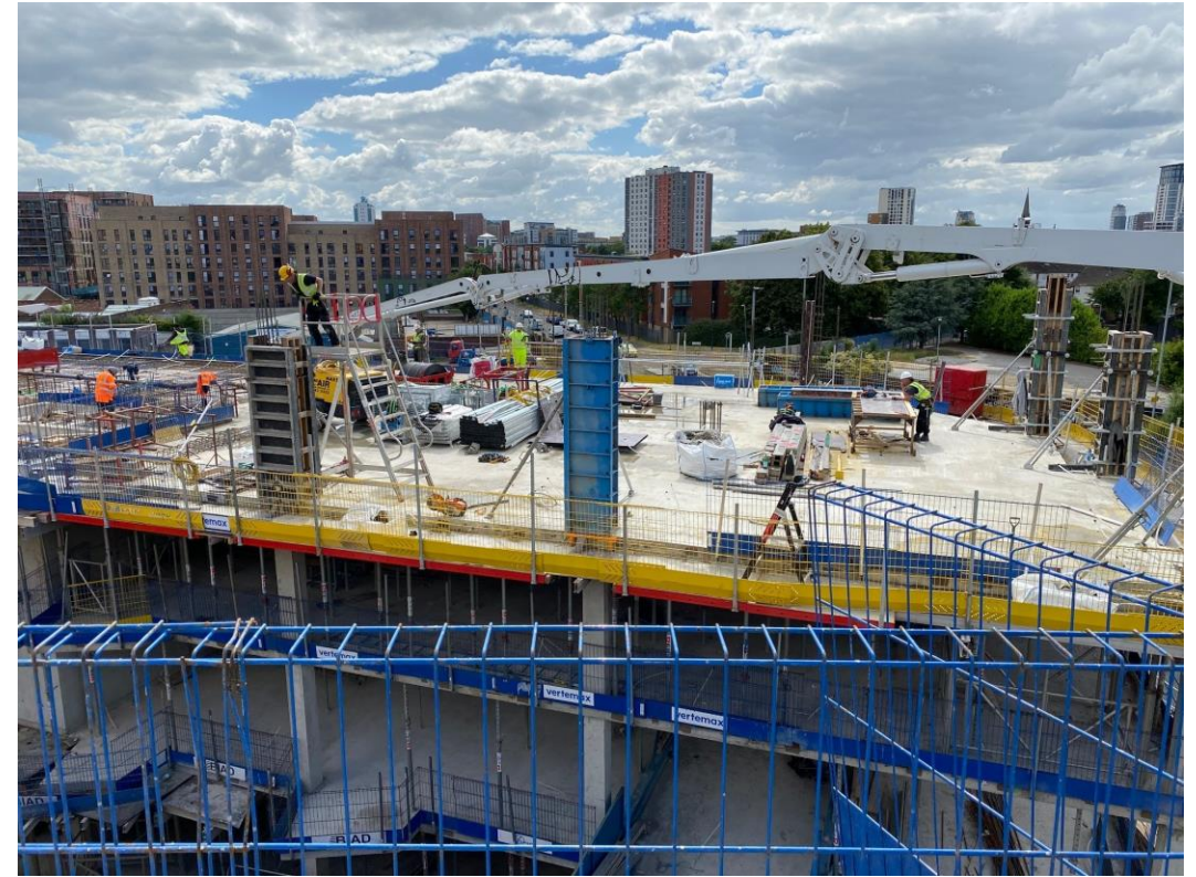
Block A concrete frame under construction
