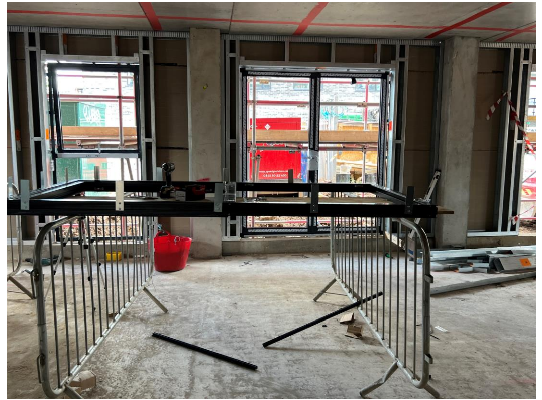
Block B ground floor window preparation
