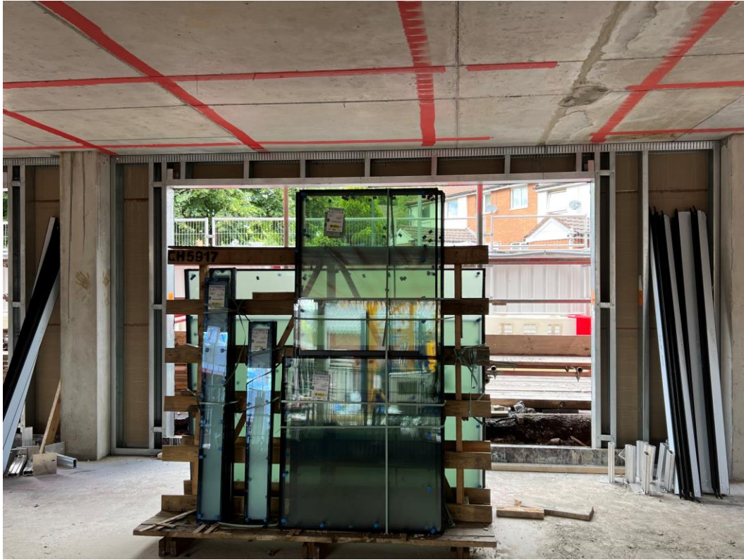
Block B ground floor windows glazing stored
