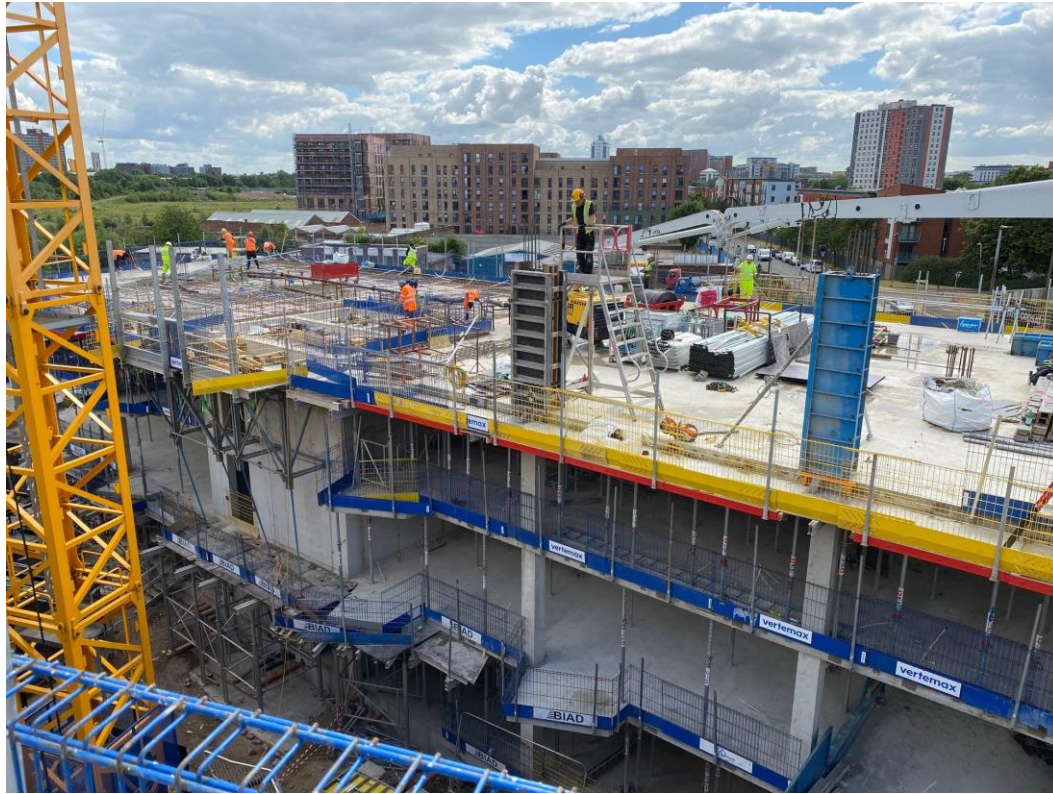
Block A concrete frame under construction
