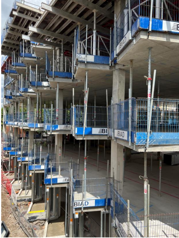
Block B concrete framework
