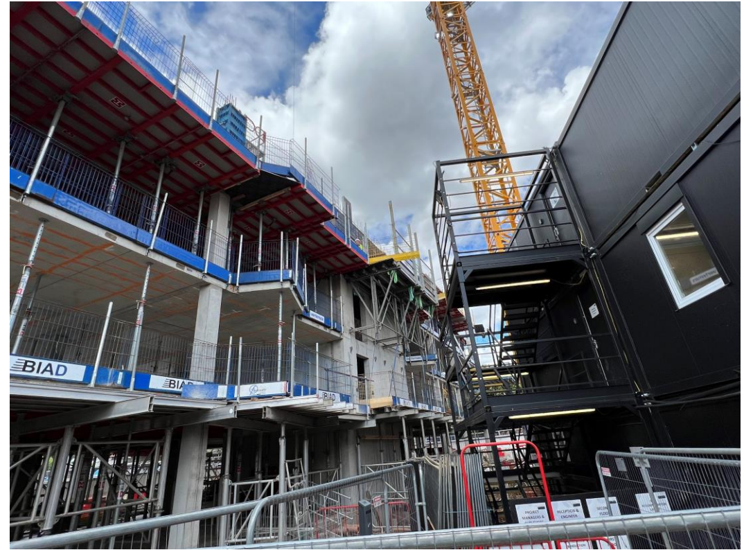
Block A concrete framework
