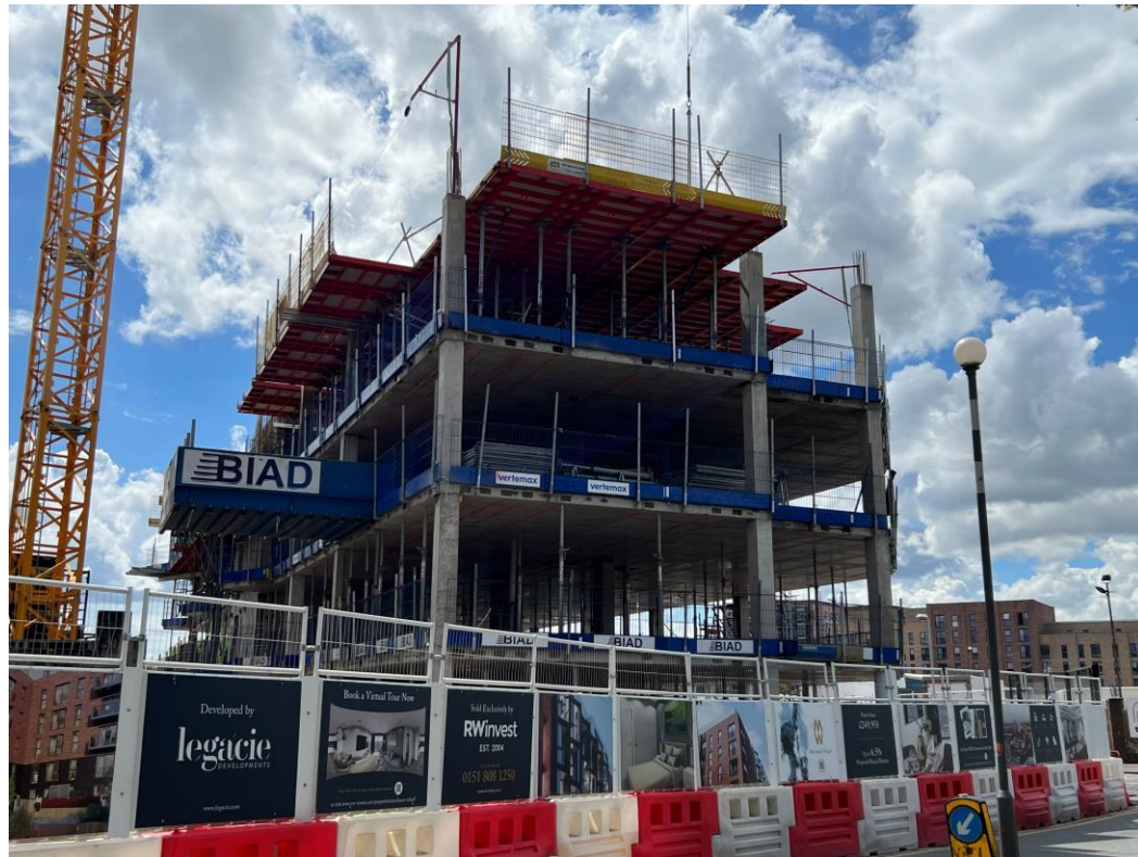
Ordsall Lane site view
