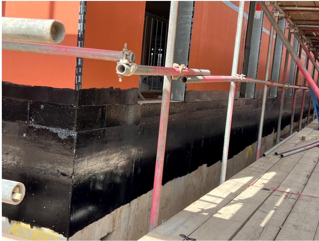
Block B SFS weatherboarding & tanking
