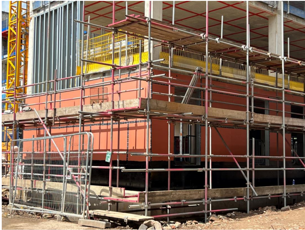
Block B SFS & weatherboarding
