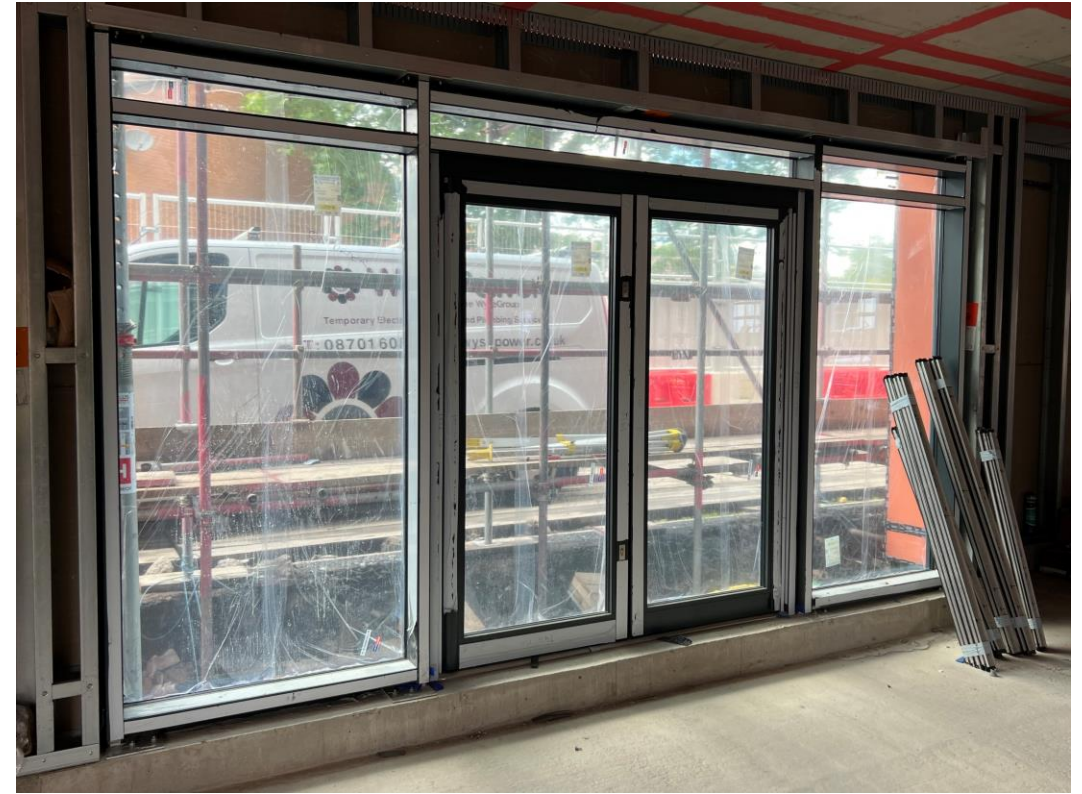
Block B ground floor windows installed
