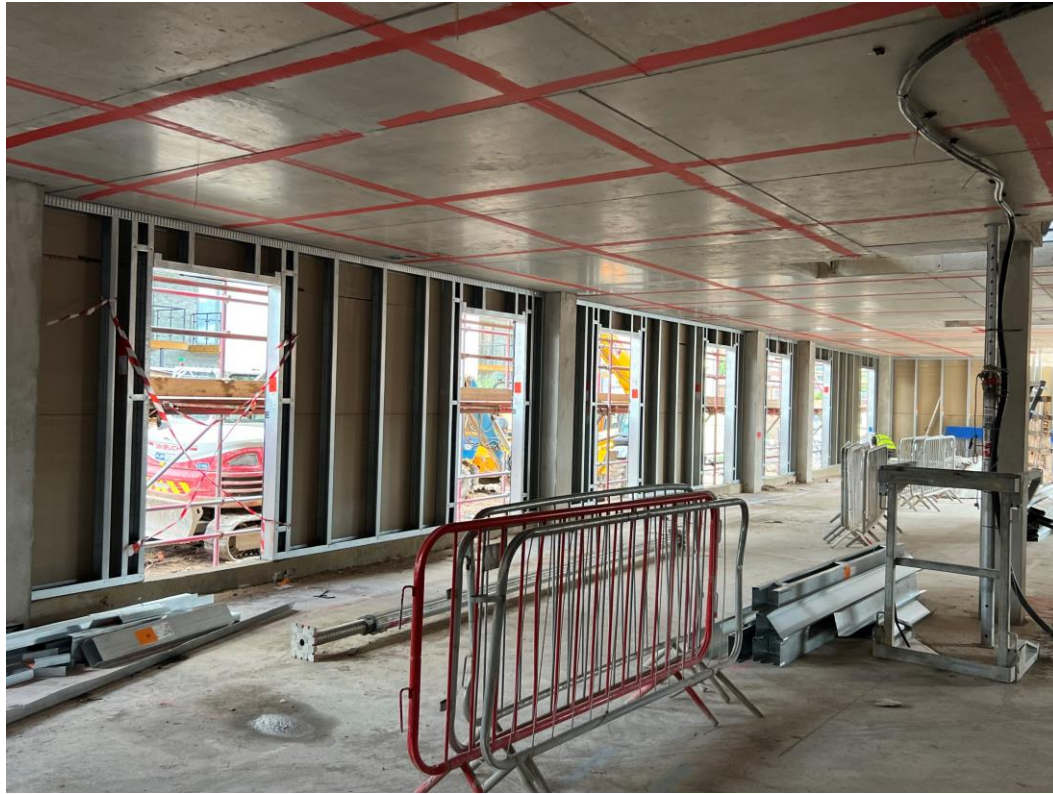
Block B ground floor SFS & weatherboarding
