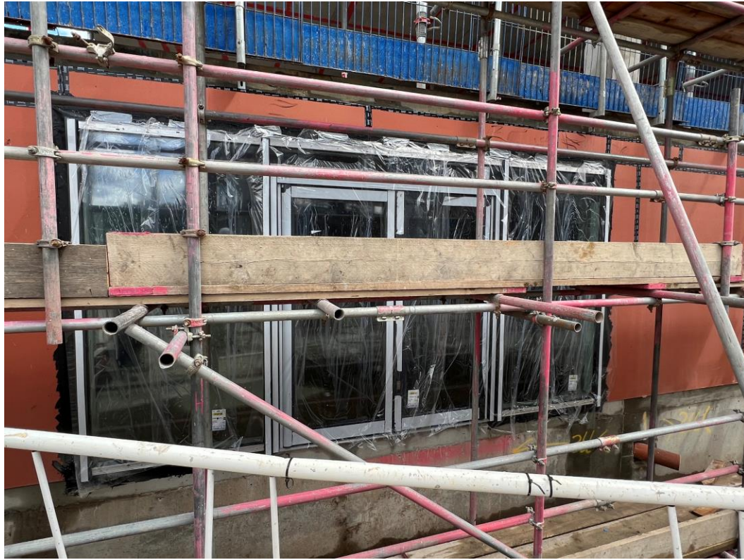
Block B external windows & doors
