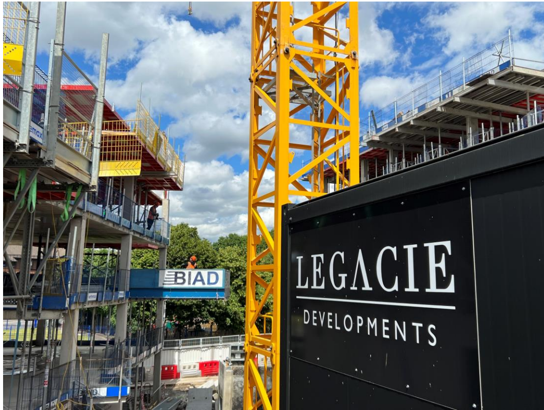
Block A concrete framework
