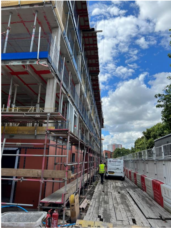
Block B SFS & weatherboarding
