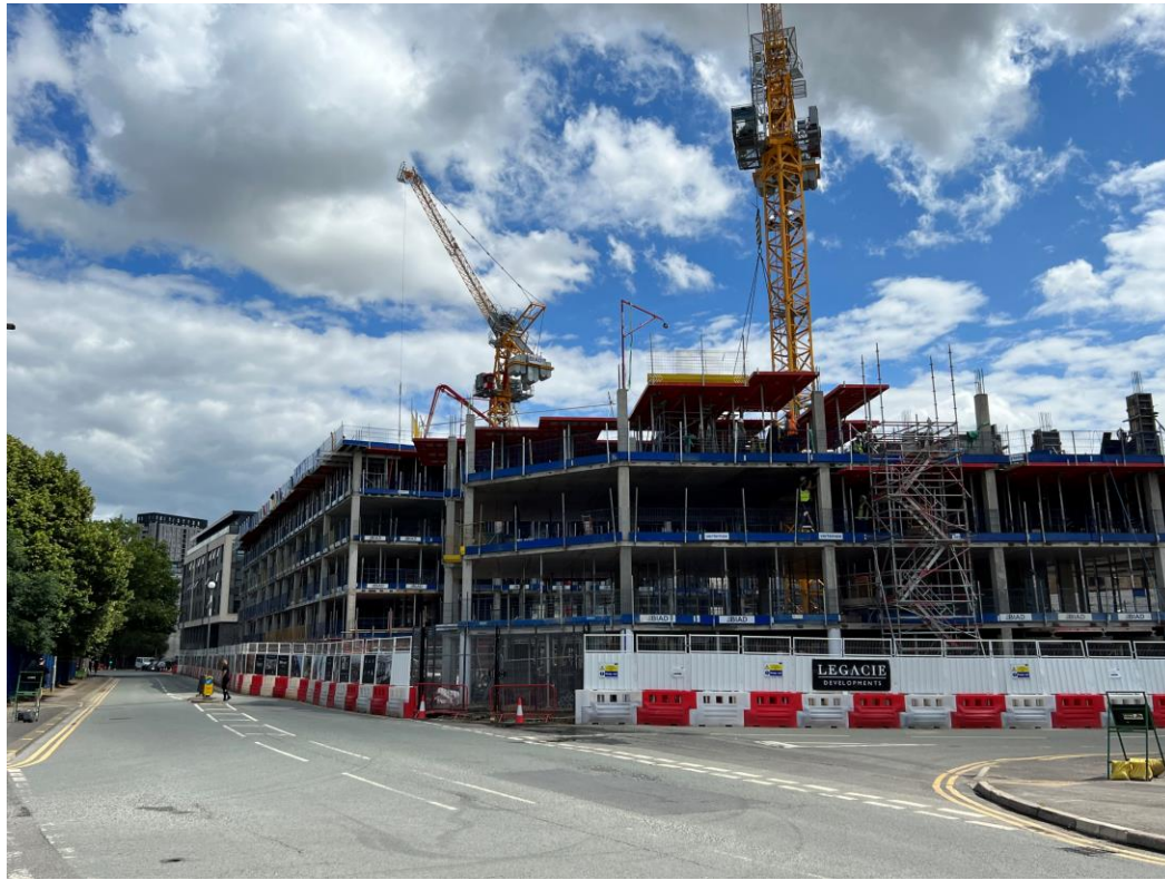
Ordsall Lane site view
