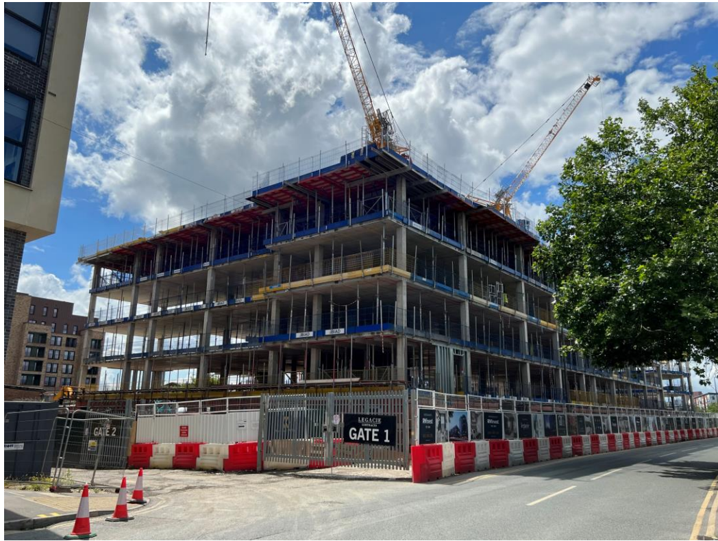
Ordsall Lane site view
