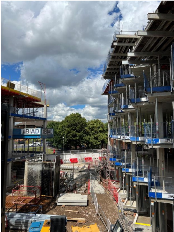
Block A & B concrete framework
