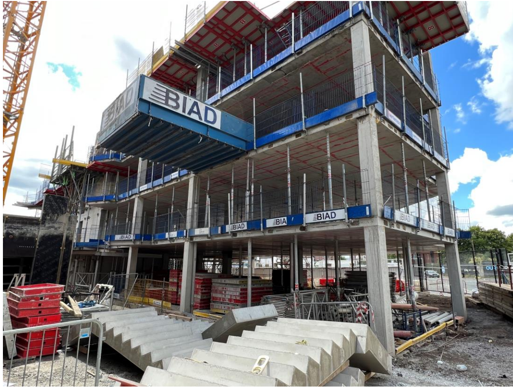
Block A concrete framework
