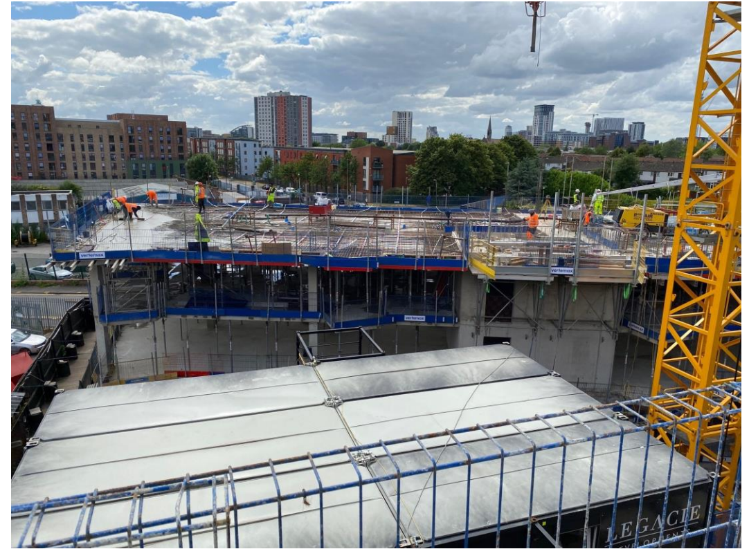
Block B concrete frame under construction
