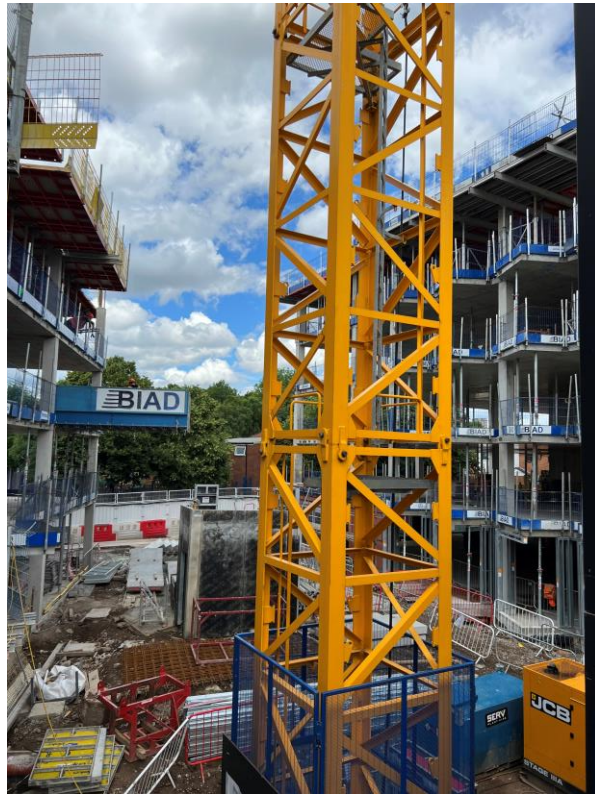
Block A & B concrete framework
