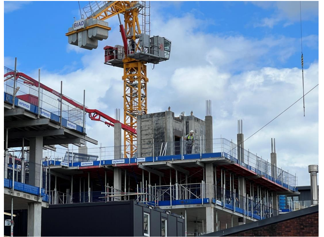
Worrall Street site view
