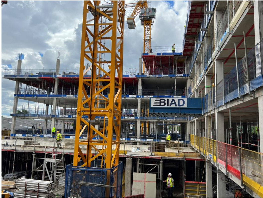
Block B concrete framework
