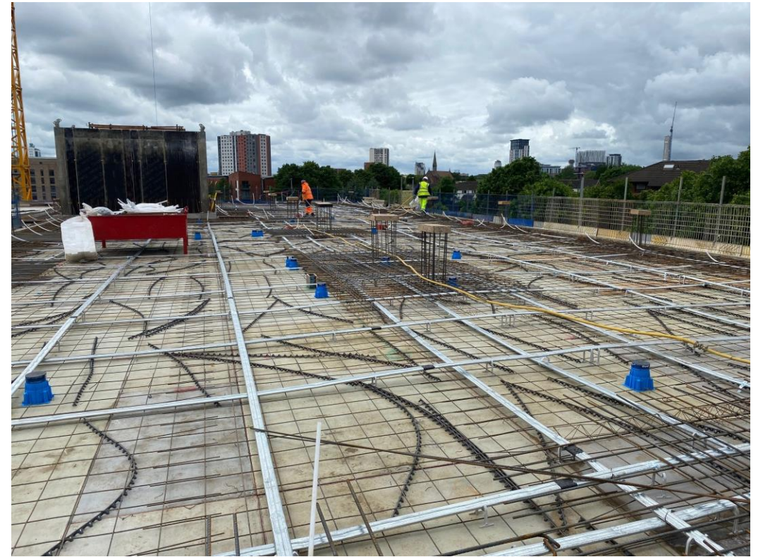
Block B concrete PT slab & column structure
