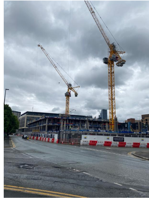
Ordsall Lane site view
