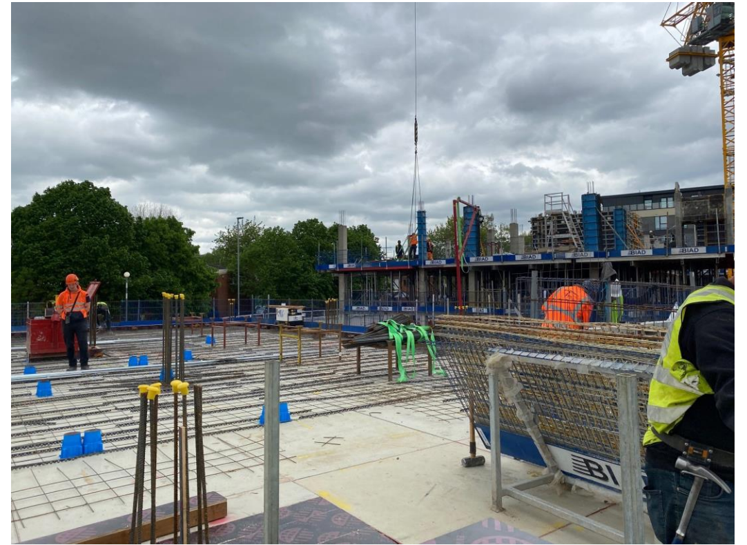
Block A upper floor slab and columns
