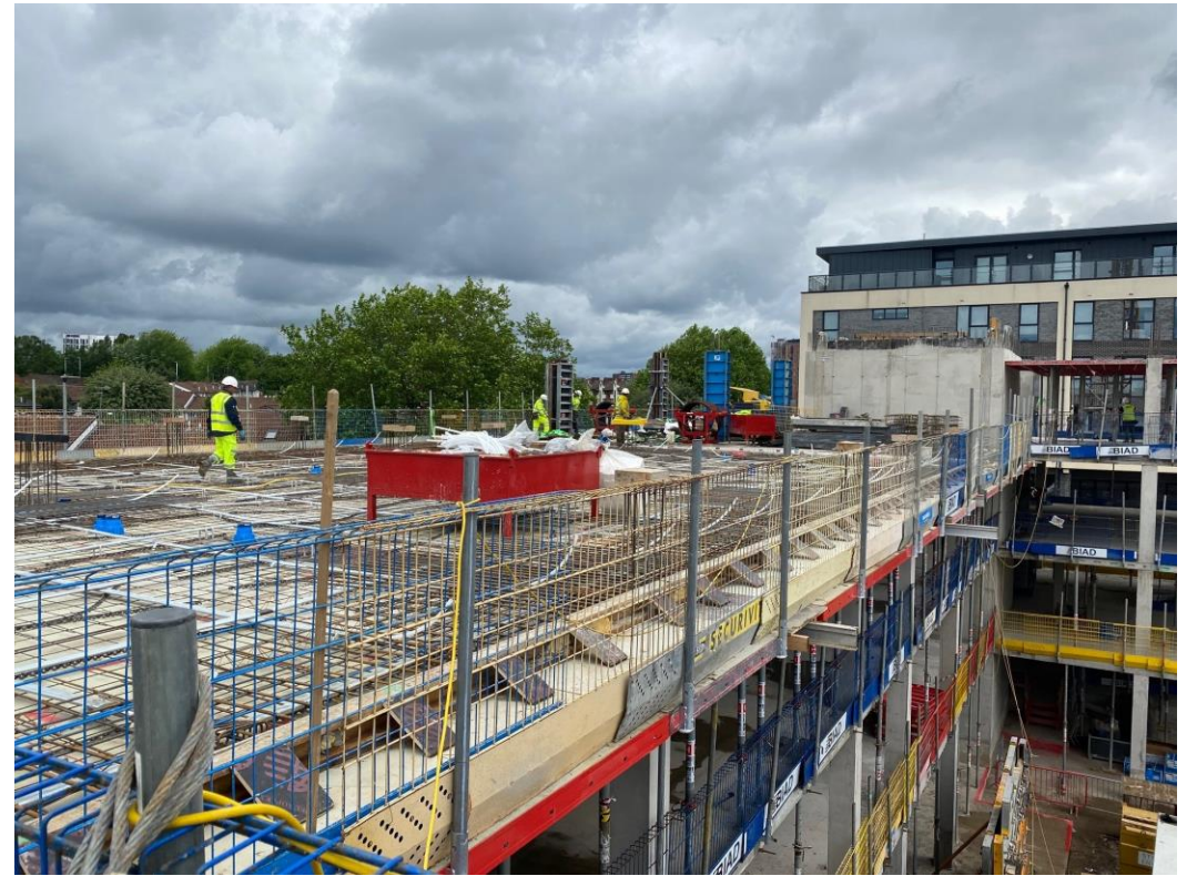
Block B sub-structure
