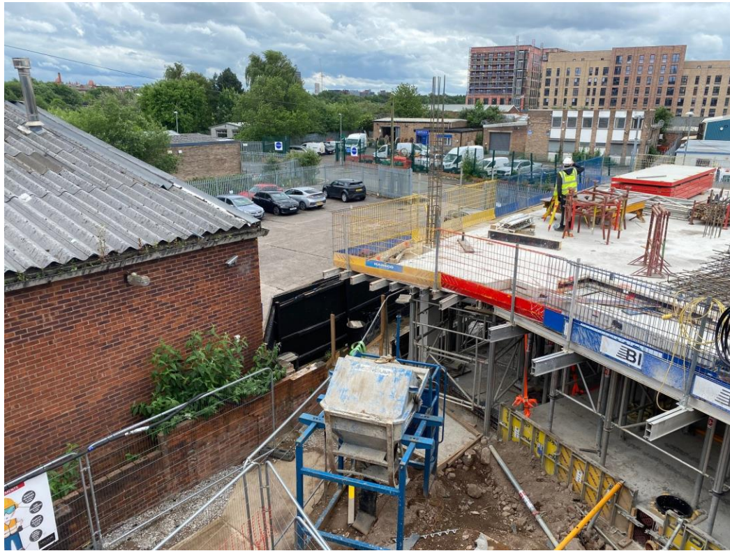
Block A upper floor slab and columns
