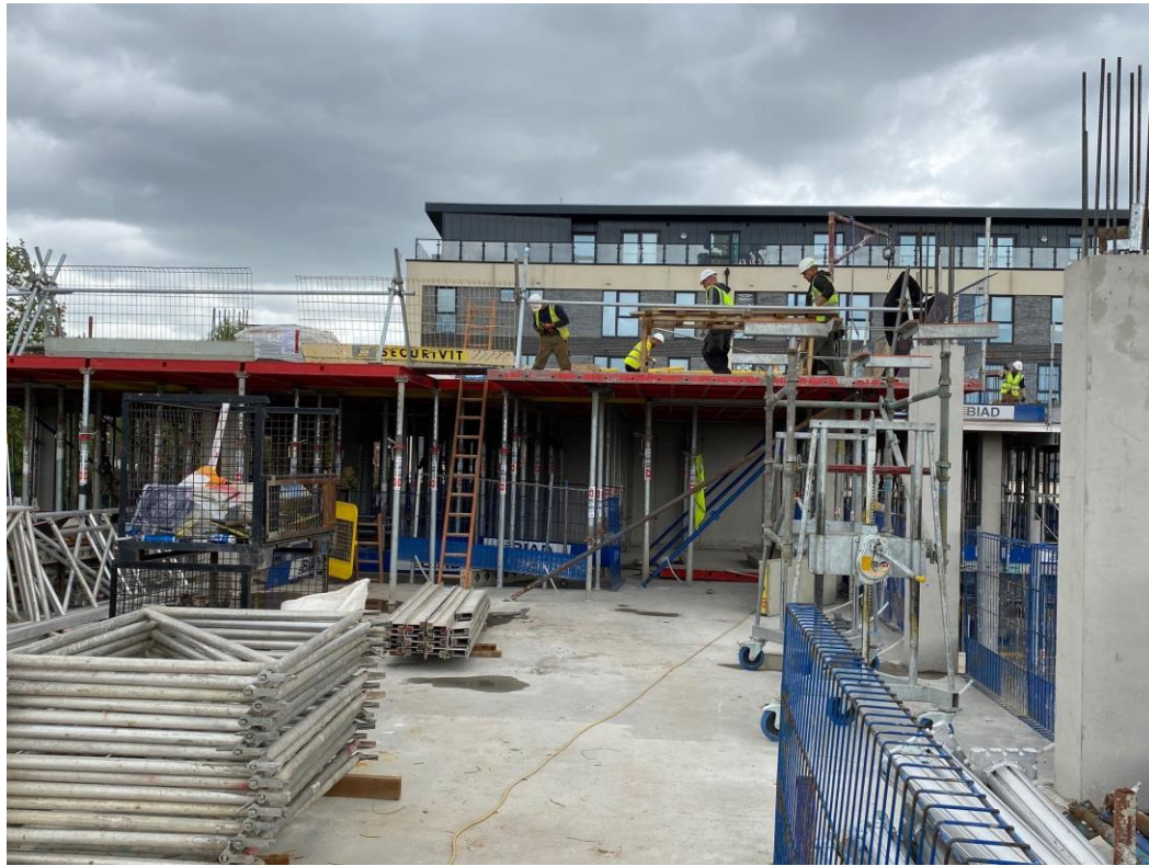
Block B upper floor slab and columns
