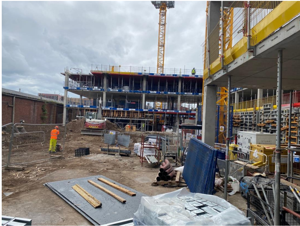
Block B upper floor slab and columns
