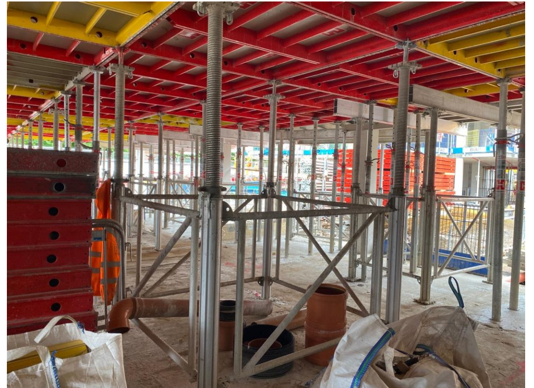
Block B Shuttering
