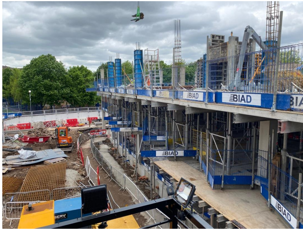
Block B upper floor slab and columns
