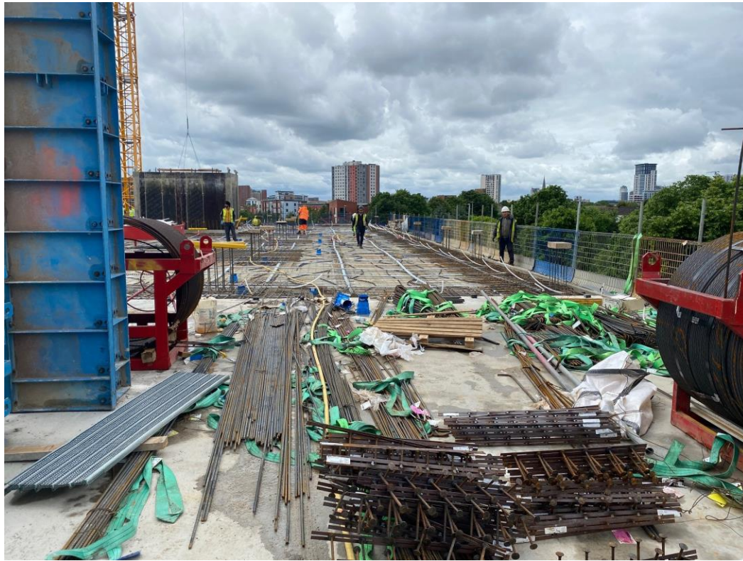
Block B concrete PT slab & column structure
