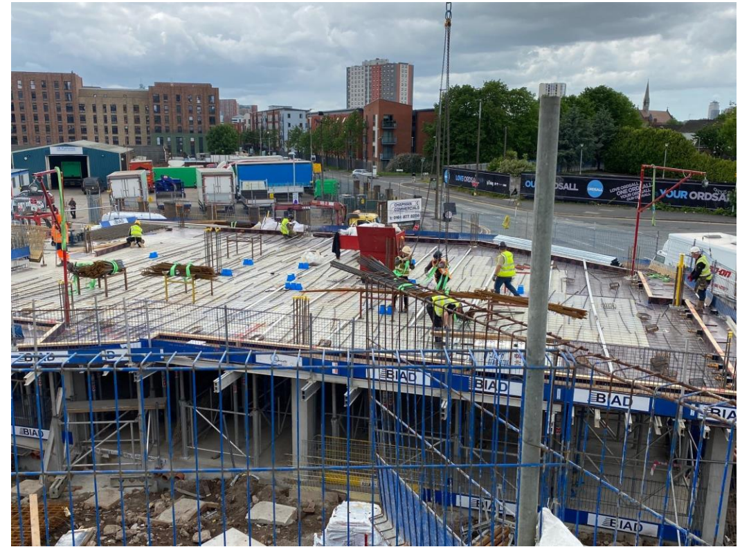
Block A upper floor slab and columns
