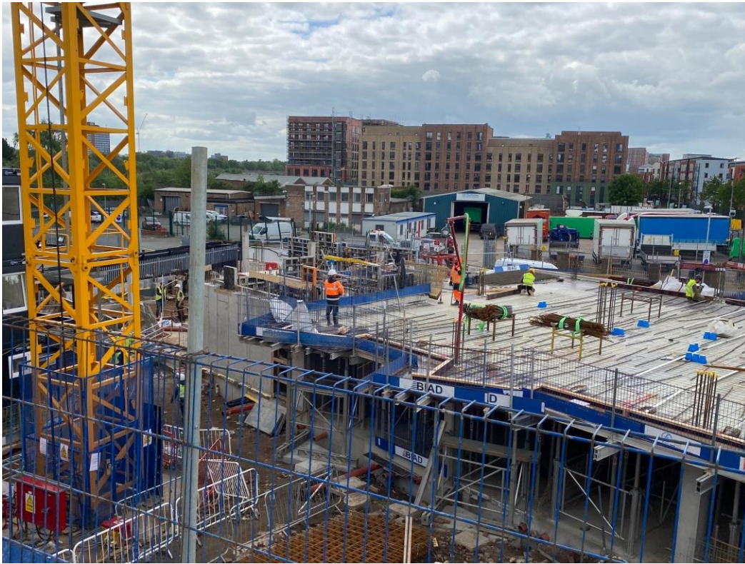
Block A upper floor slab and columns
