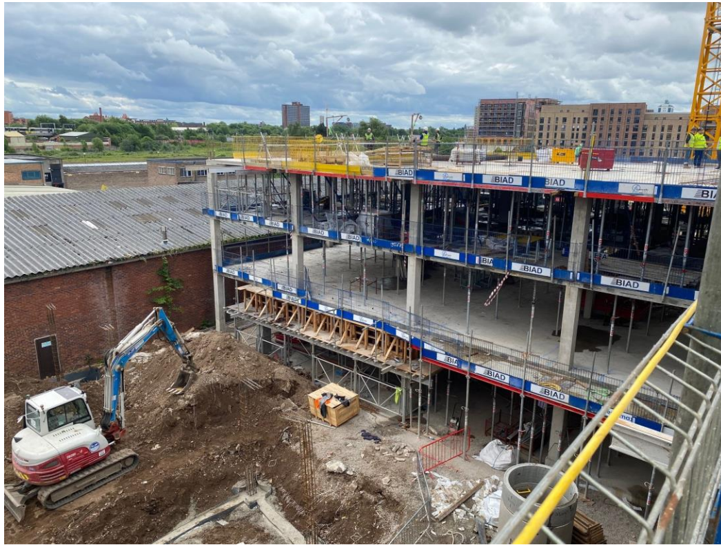
Block B upper floor slab and columns
