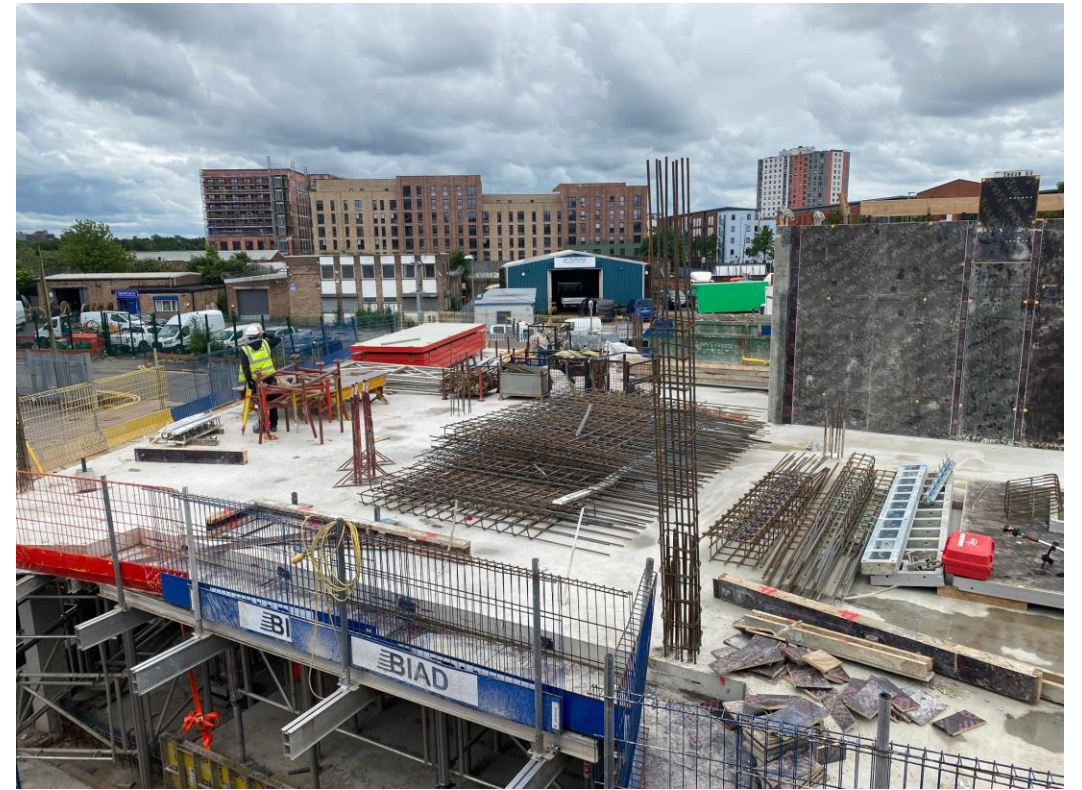
Block A upper floor slab and columns
