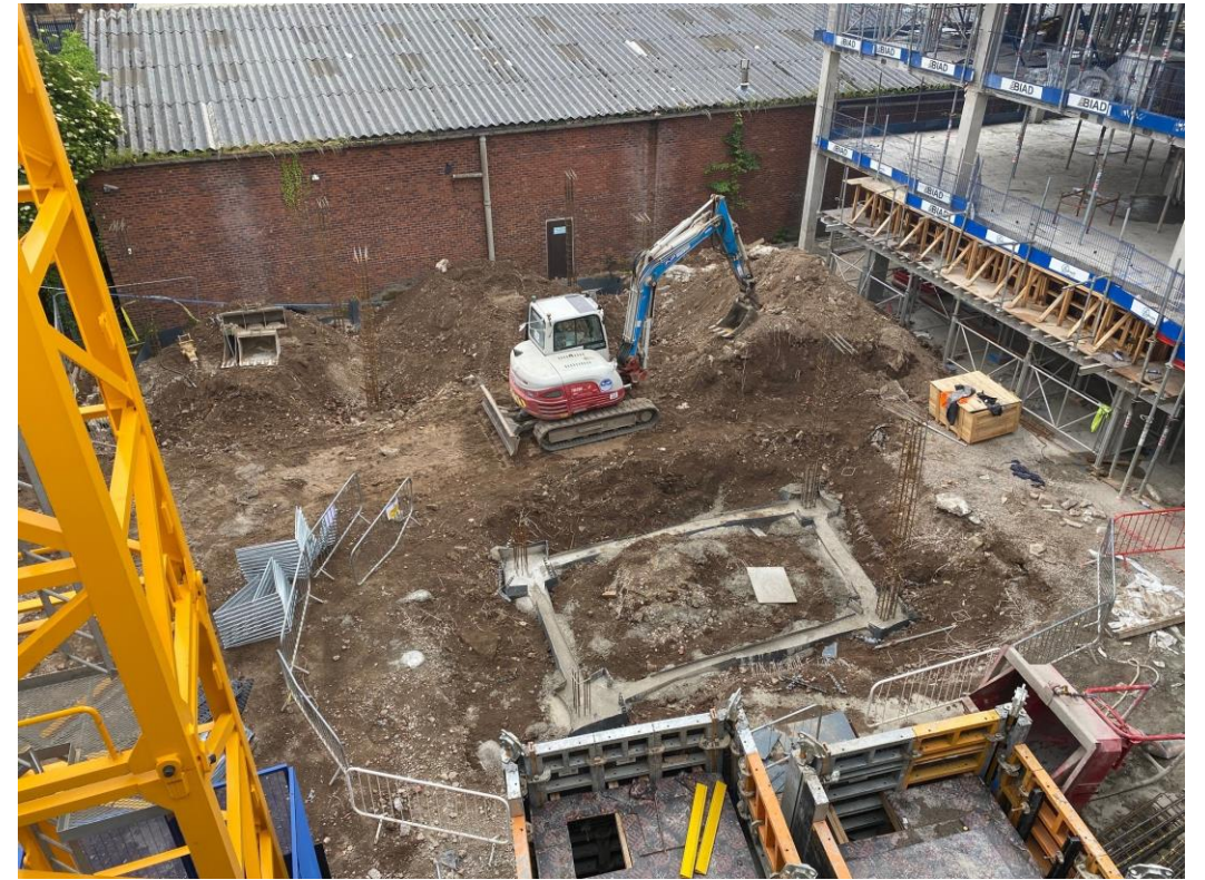
Block B sub-structure
