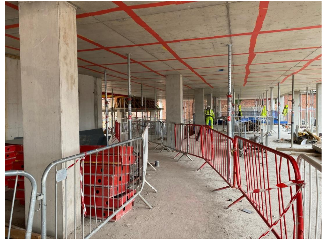
Block B superstructure
