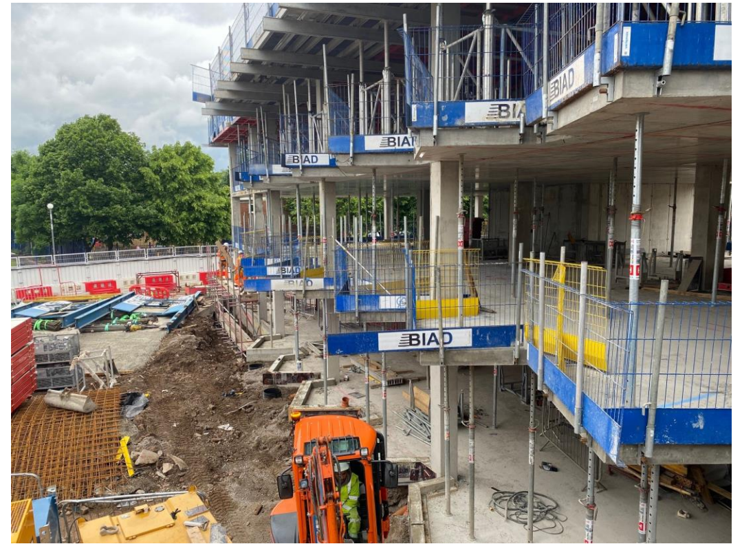
Block B upper floor slab and columns
