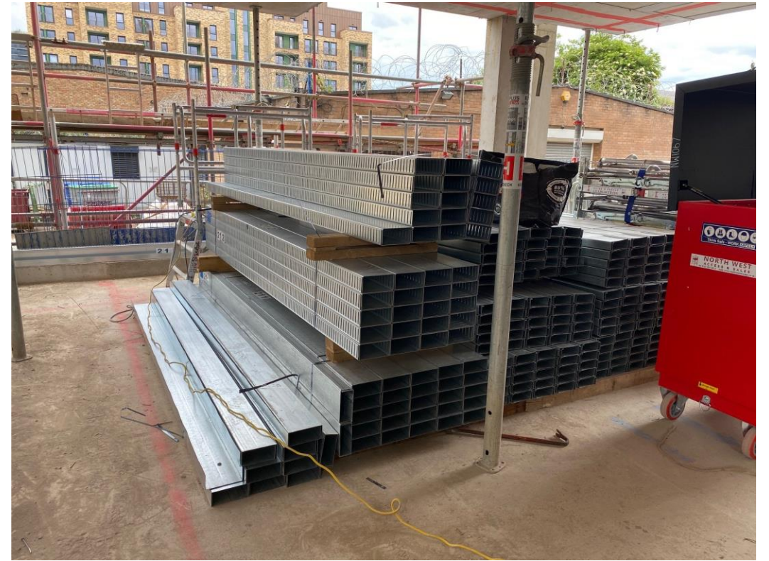
Block B sfs material storage
