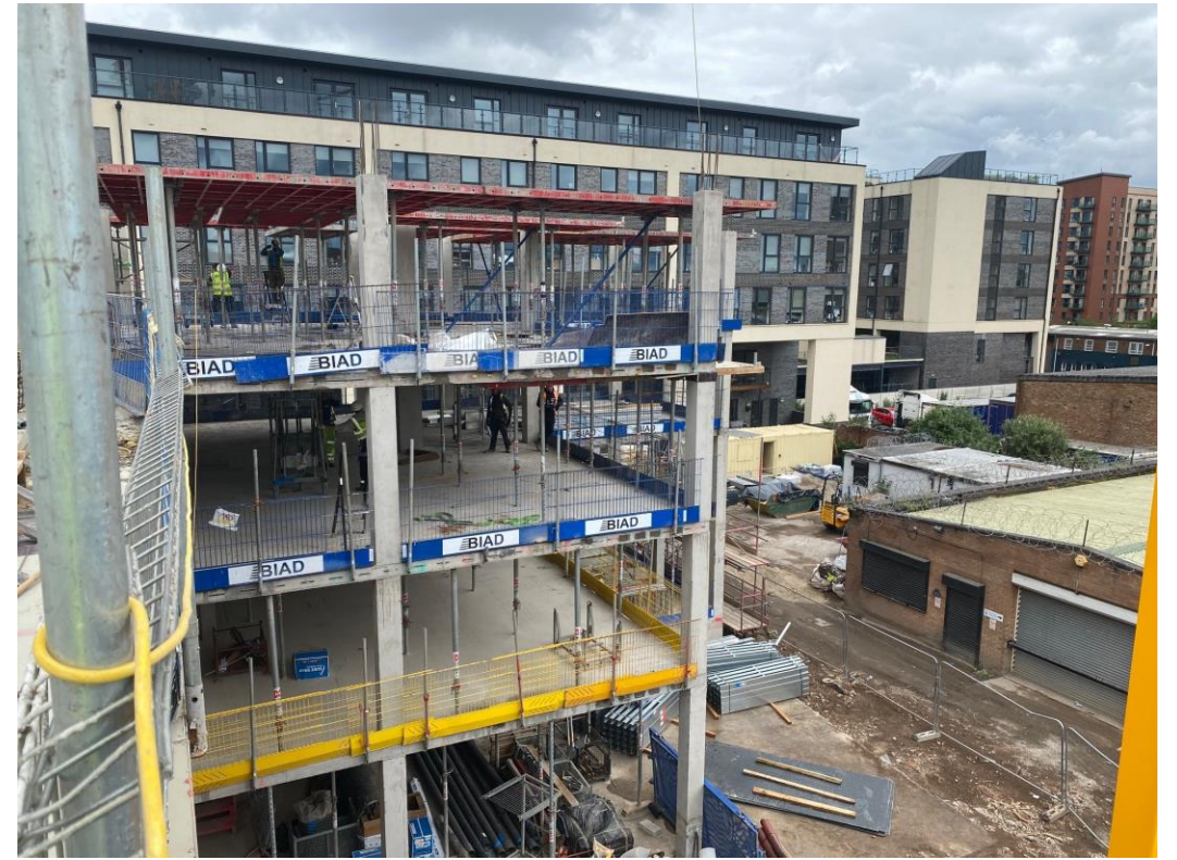
Block B upper floor slab and columns
