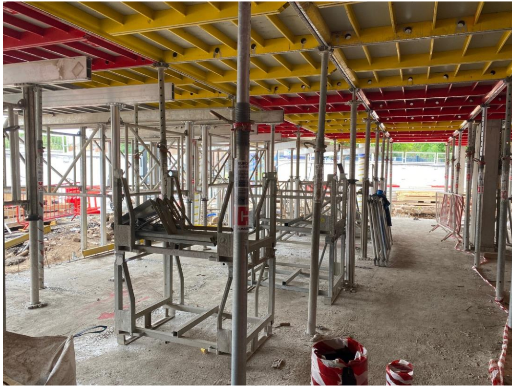
Block B Shuttering
