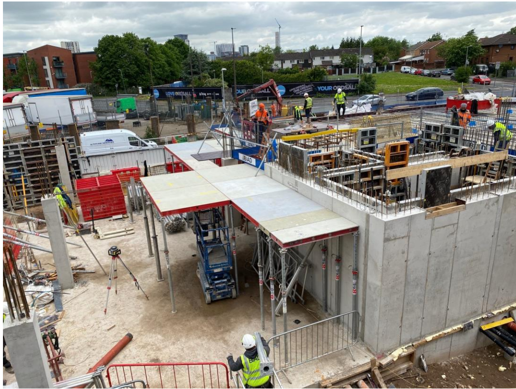
Block A upper floor slab and columns
