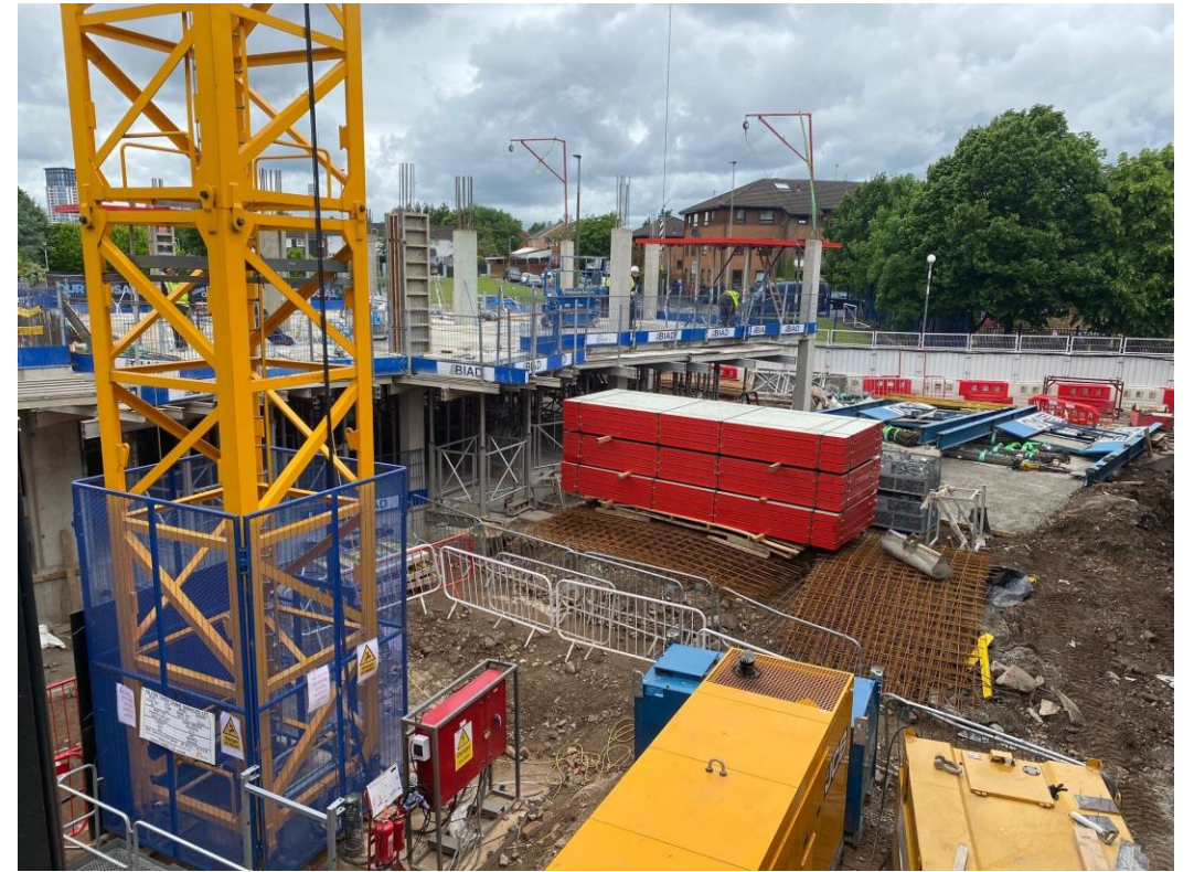
Block A upper floor slab and columns
