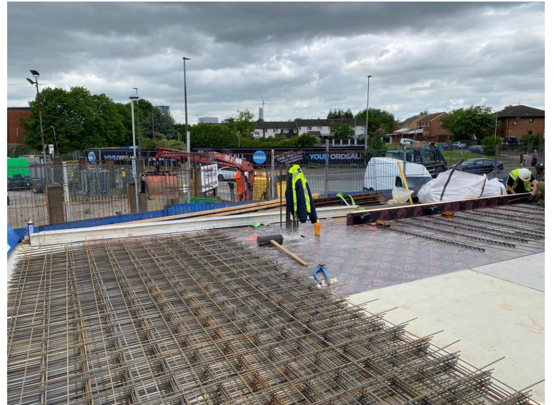
Block A upper floor slab and columns
