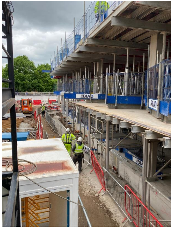
Block B upper floor slab and columns
