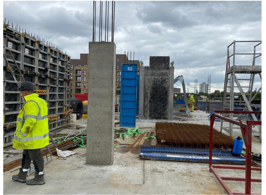
Block B upper floor slab and columns
