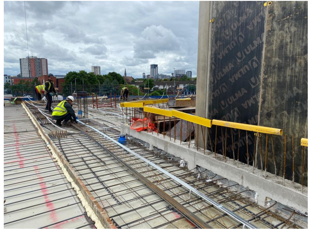
Block B concrete PT slab & column structure
