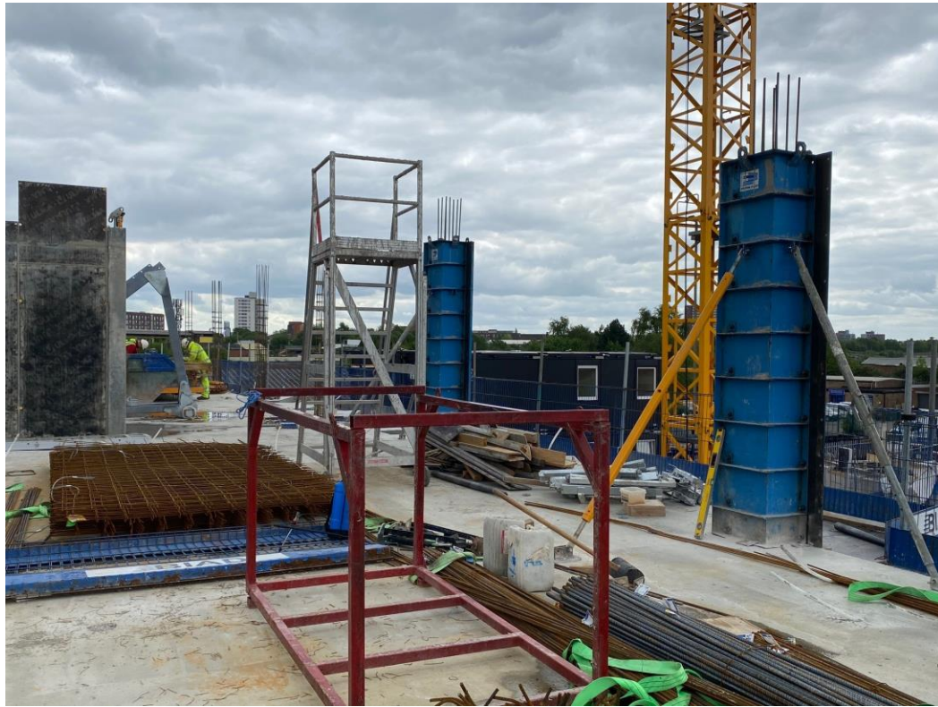
Block B upper floor slab and columns
