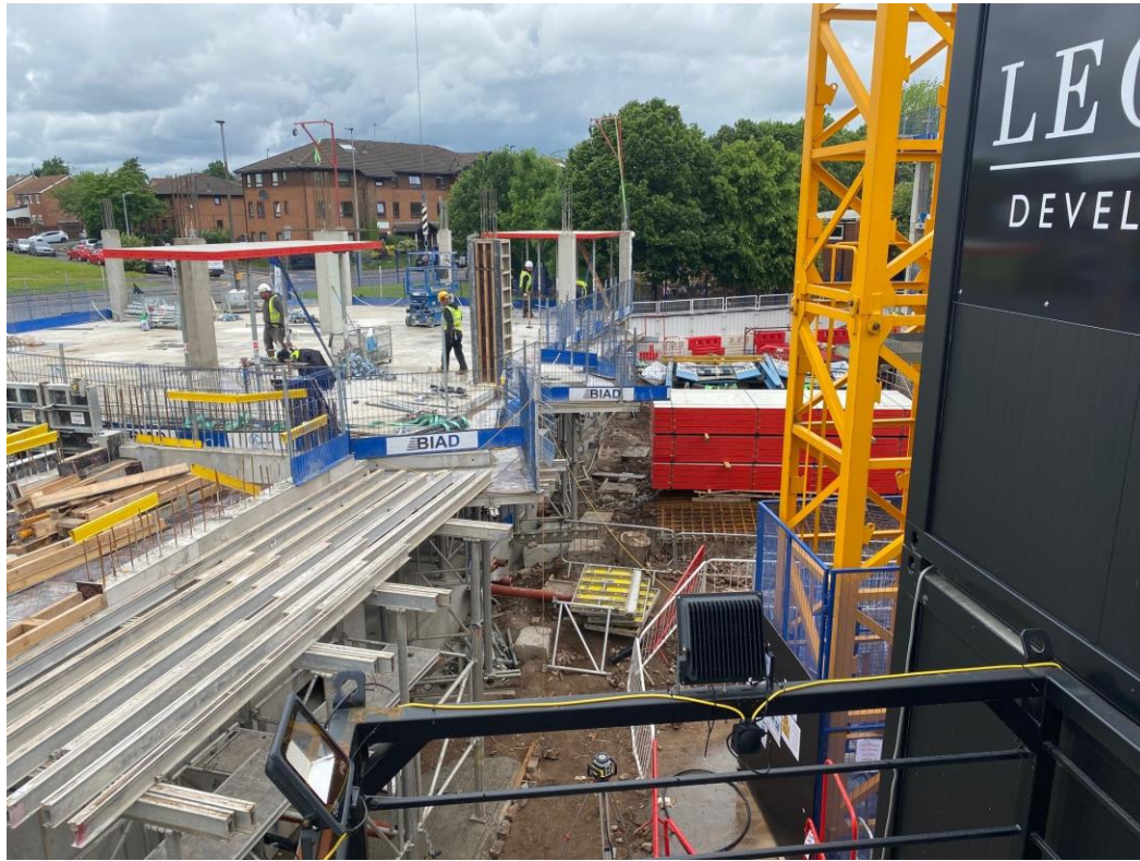
Block A upper floor slab and columns
