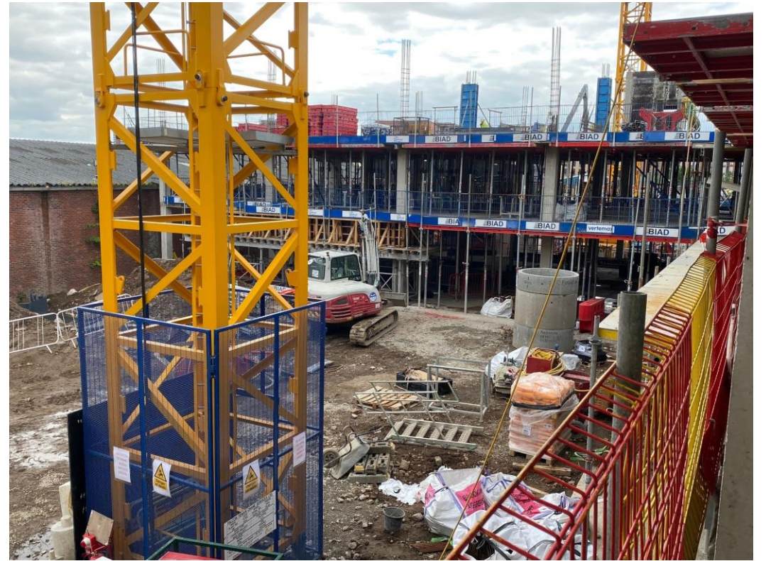
Block C upper floor slab and columns
