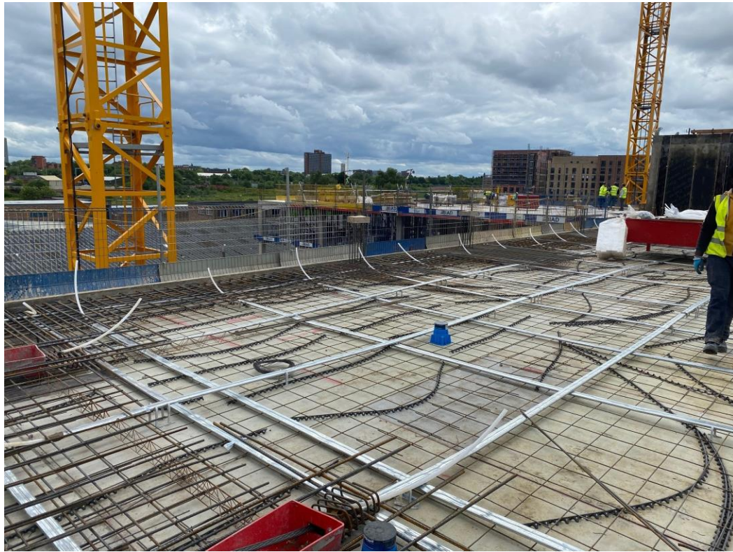
Block B concrete PT slab & column structure
