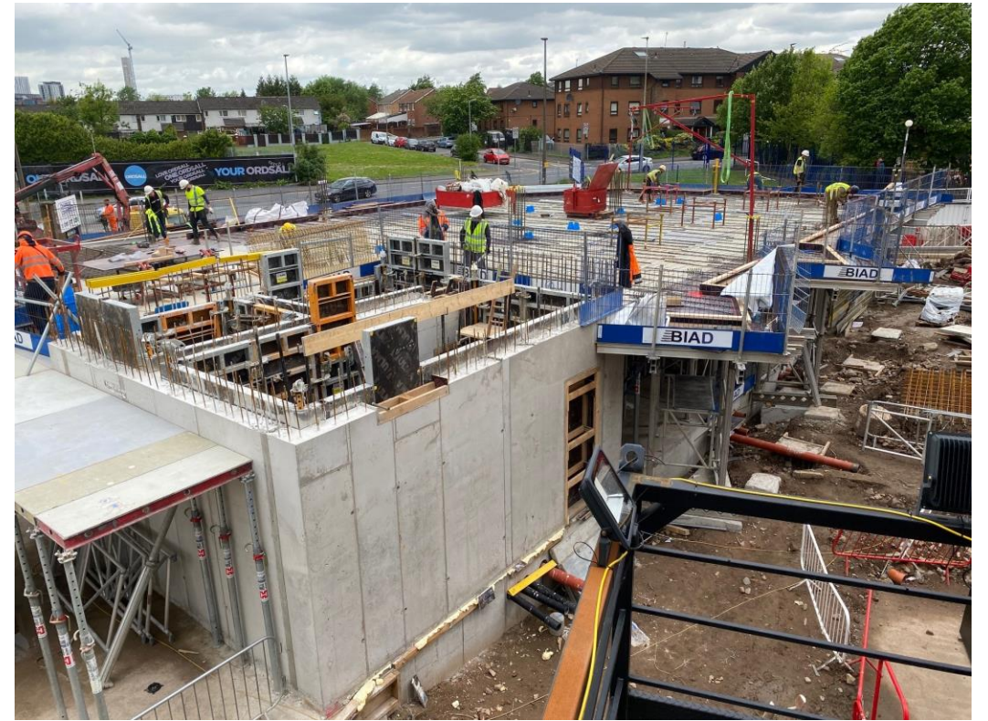
Block A upper floor slab and columns
