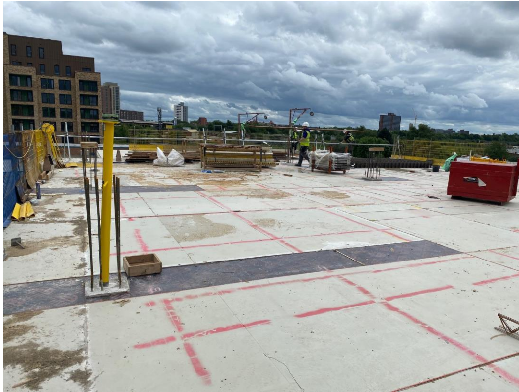
Block B concrete PT slab & column structure
