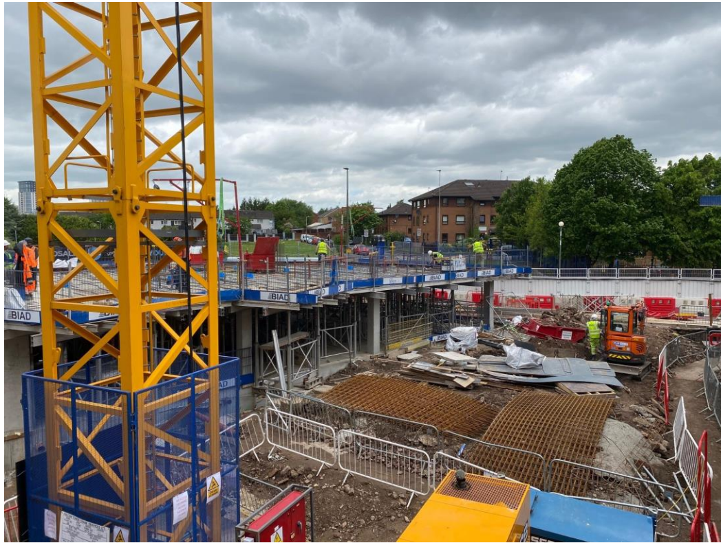
Block A upper floor slab and columns
