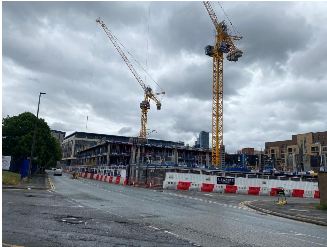
Ordsall Lane site view
