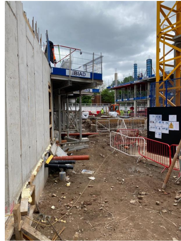
Block B drainage
