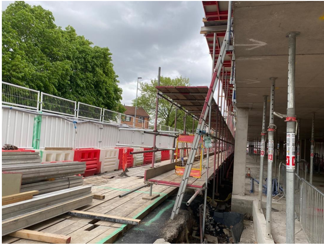
Block B scaffolding
