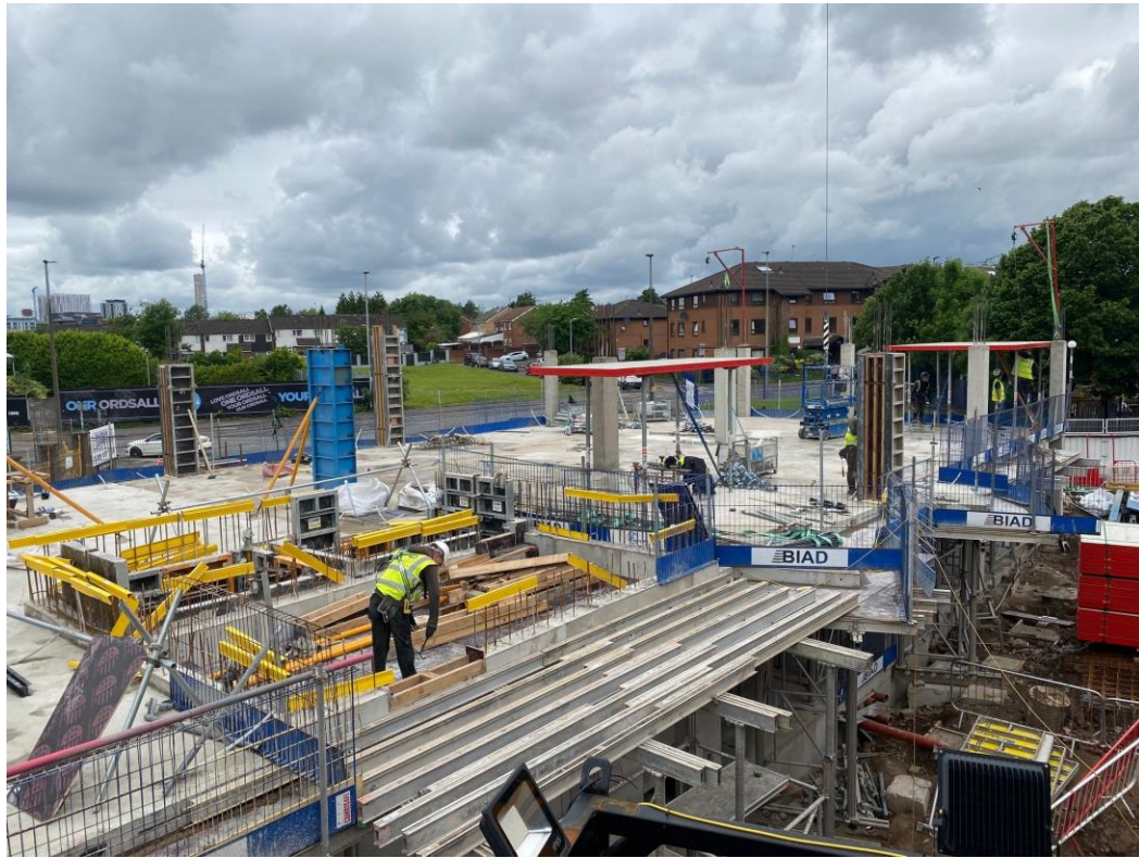
Block A upper floor slab and columns
