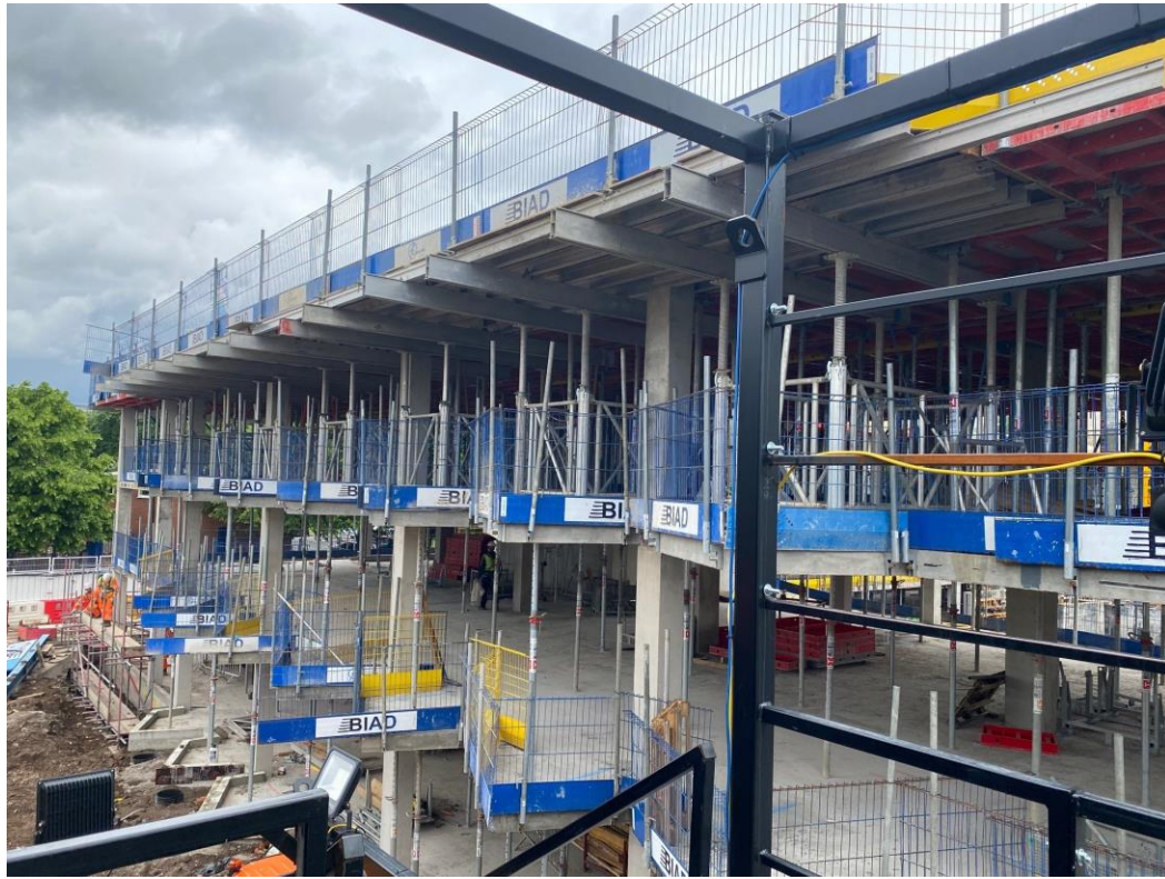
Block B upper floor slab and columns
