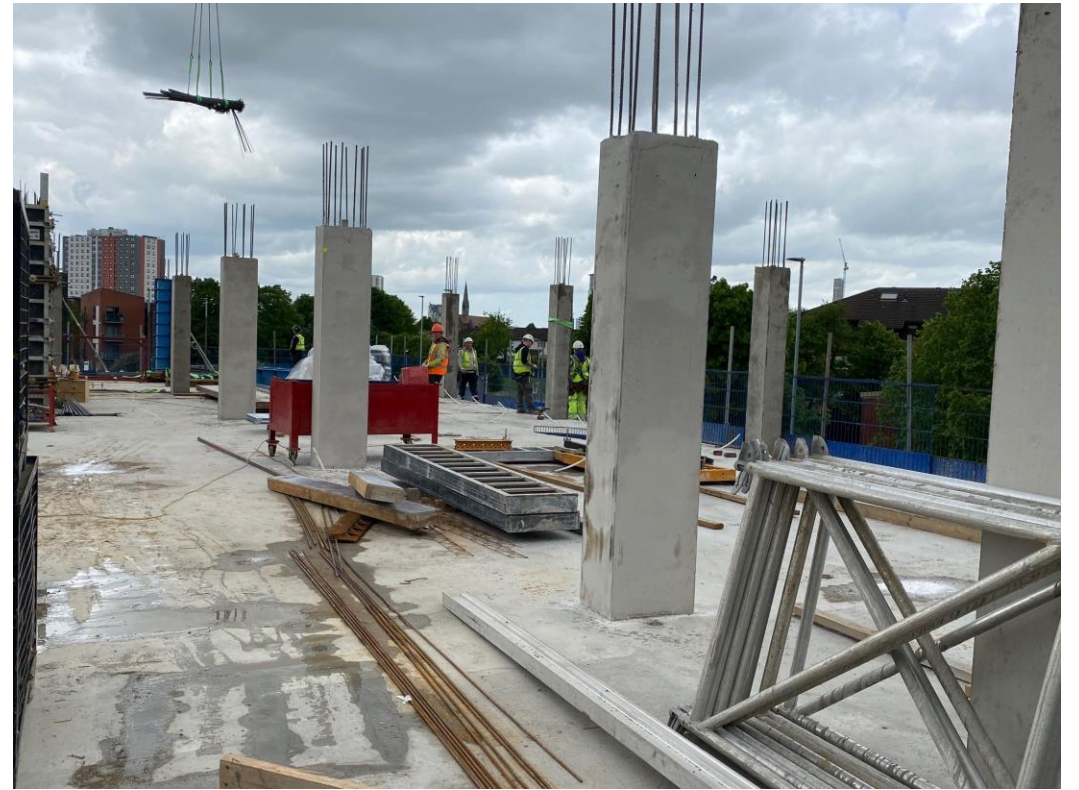
Block B upper floor slab and columns
