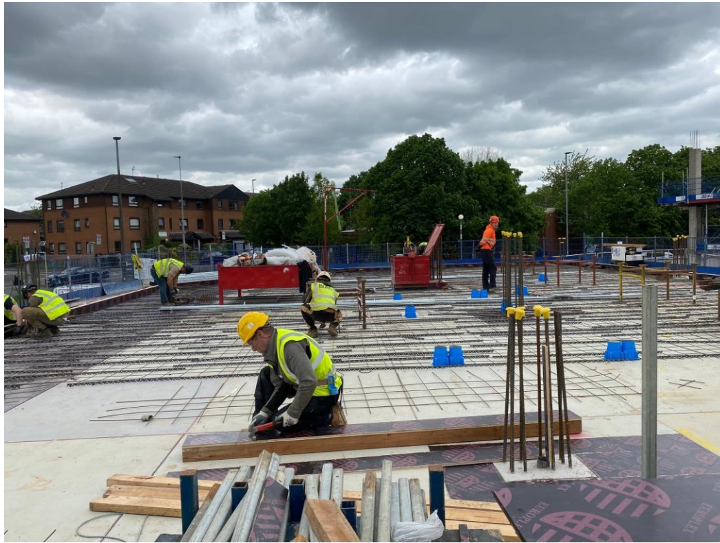
Block A upper floor slab and columns
