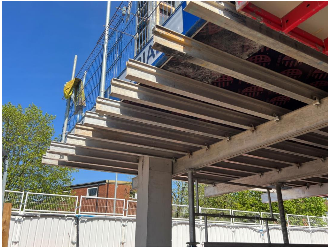
Block B superstructure
