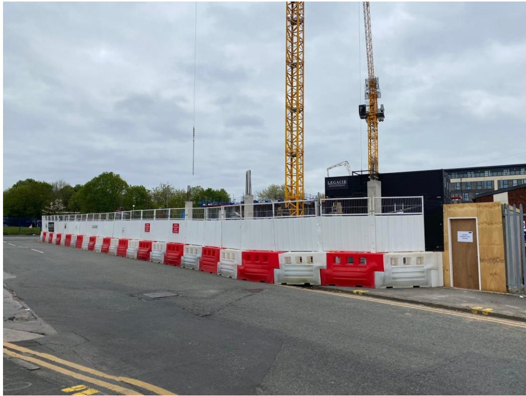
Site entrance Ordsall Lane
