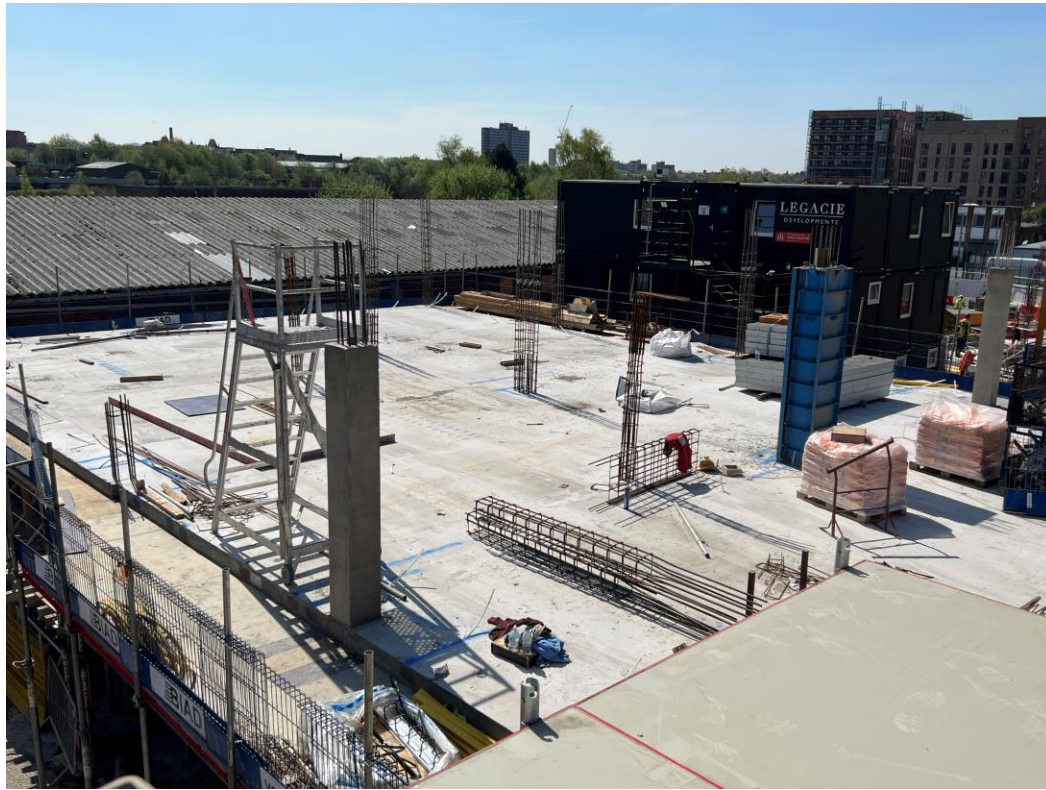
Block B First floor concrete PT slab & column structure
