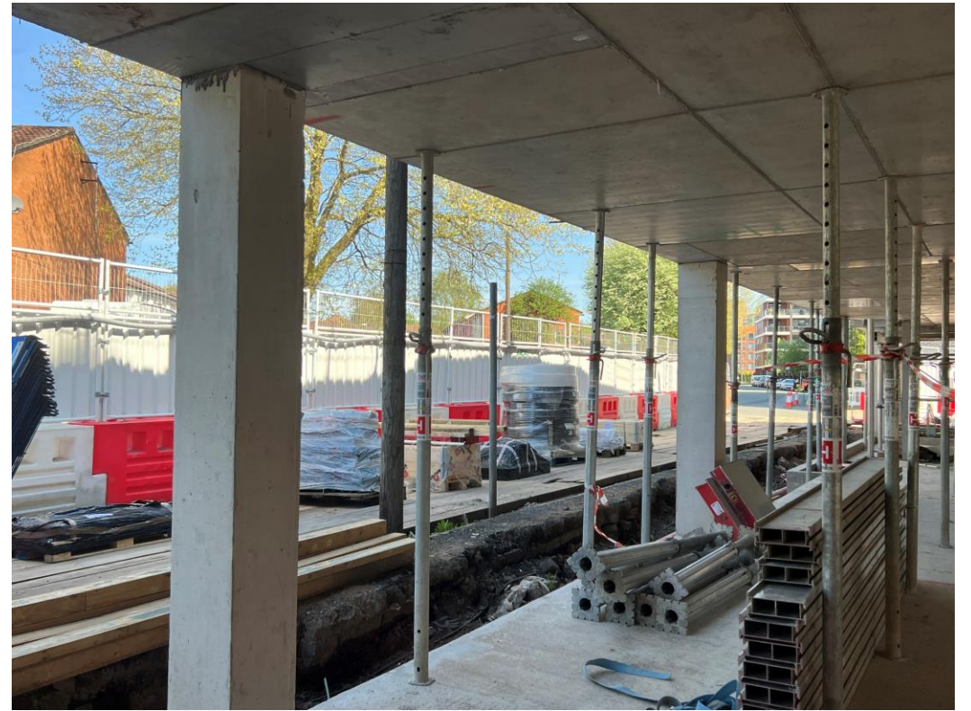
Block B superstructure
