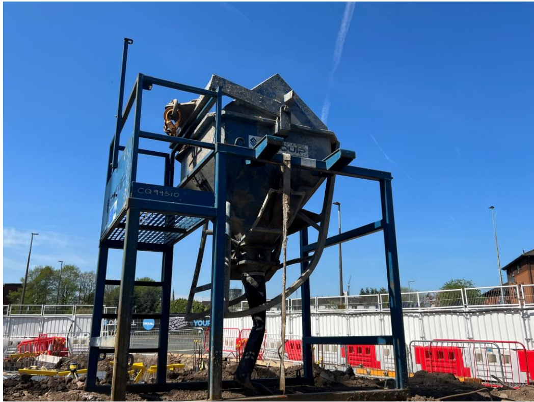
Crane lift cement bucket
