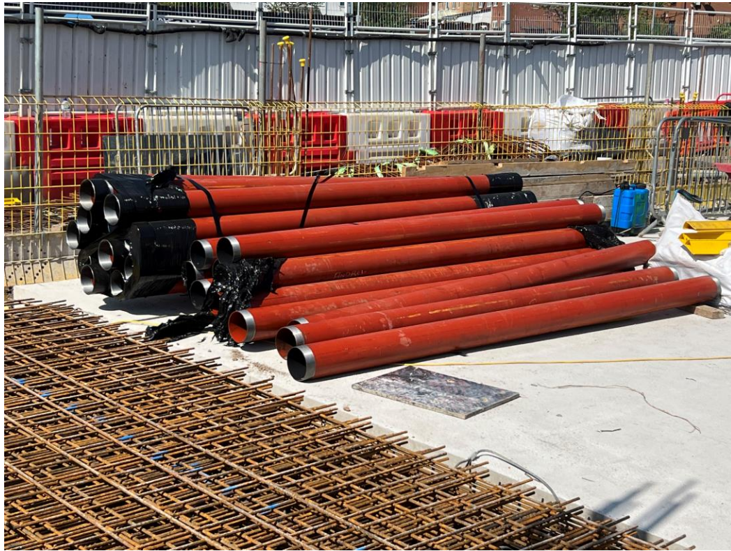
Block A underground services
