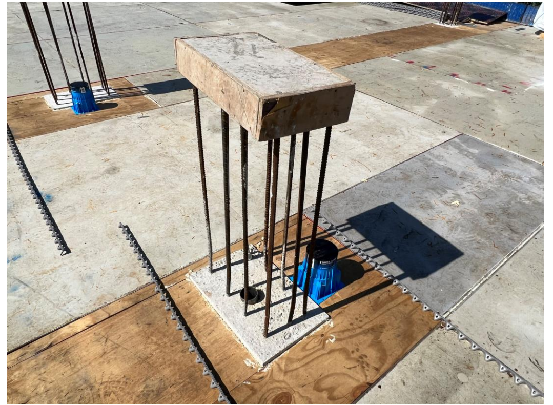
Block B PT floor slab preparation
