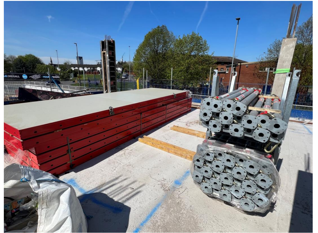
Block B shuttering materials
