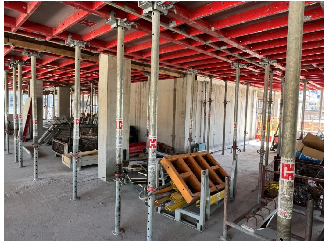
Block B lift and stair core structure
