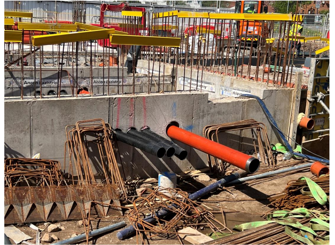
Block A underground services
