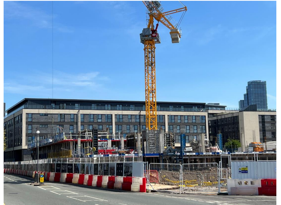
Ordsall Lane site view
