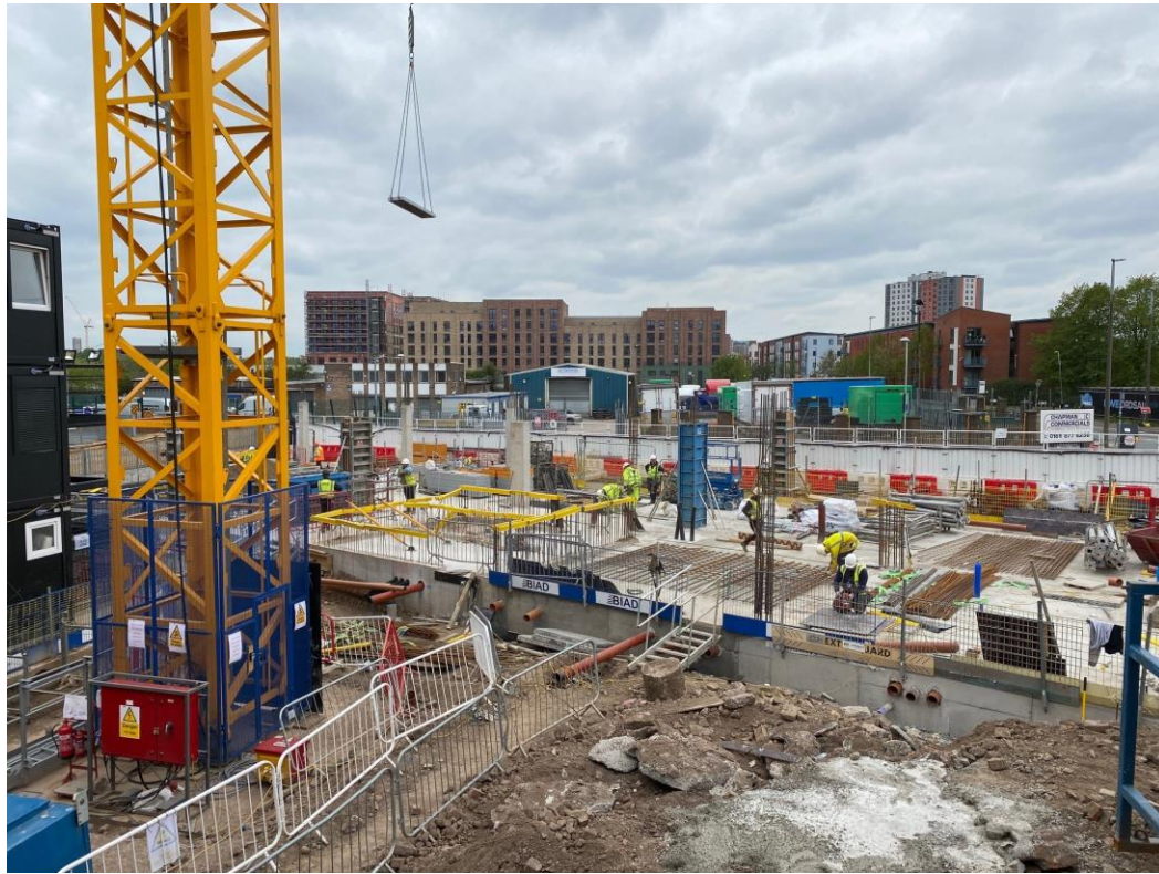
Block A site activity
