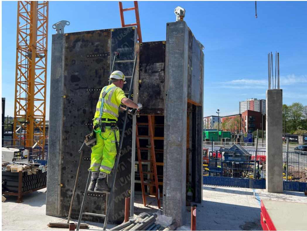
Block B lift and stair core structure
