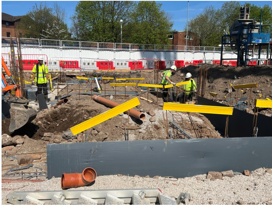
Block A substructure
