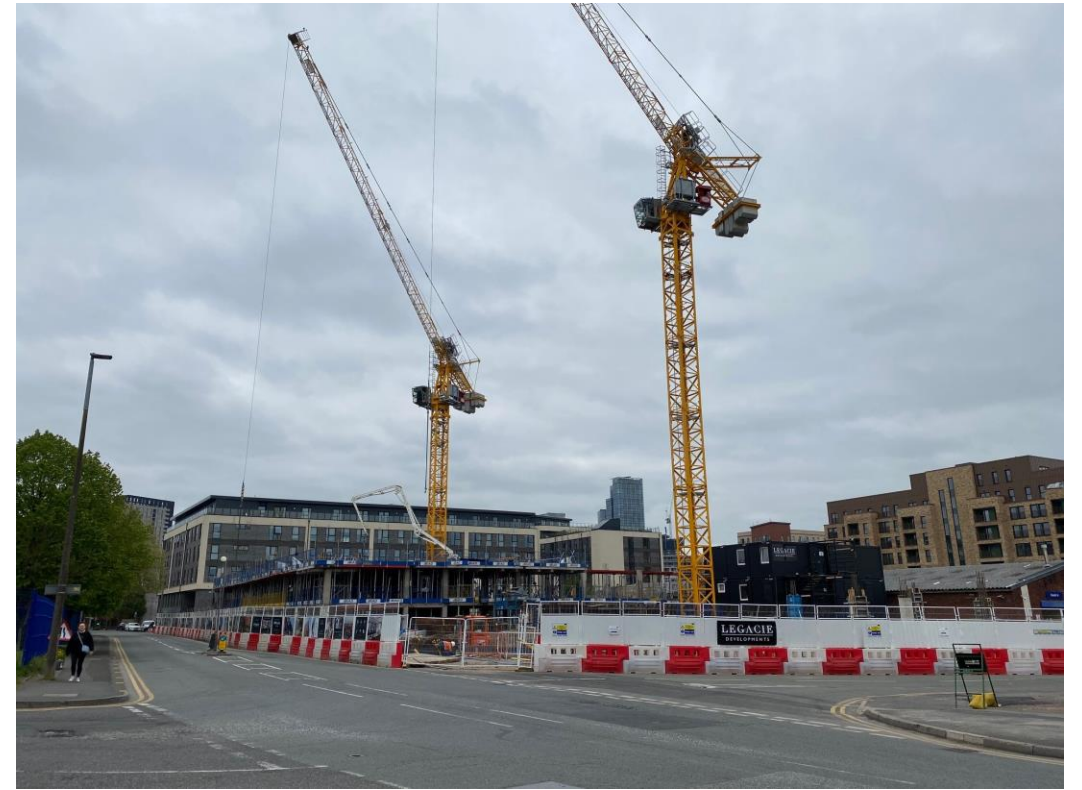
Ordsall Lane site view
