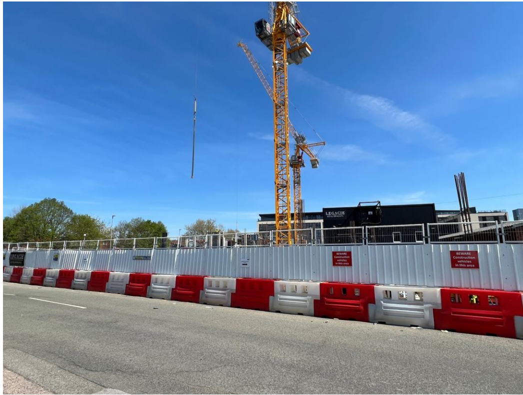
Ordsall Lane site view
