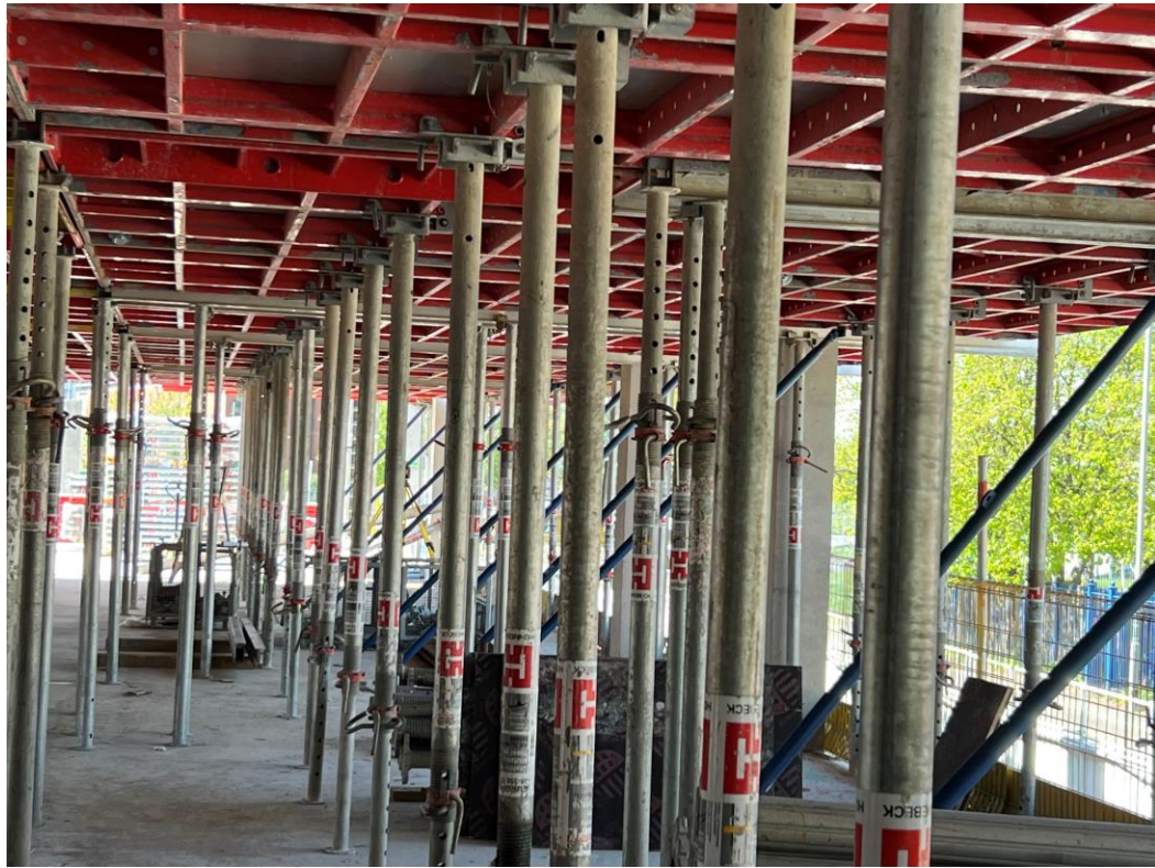
Block B Shuttering
