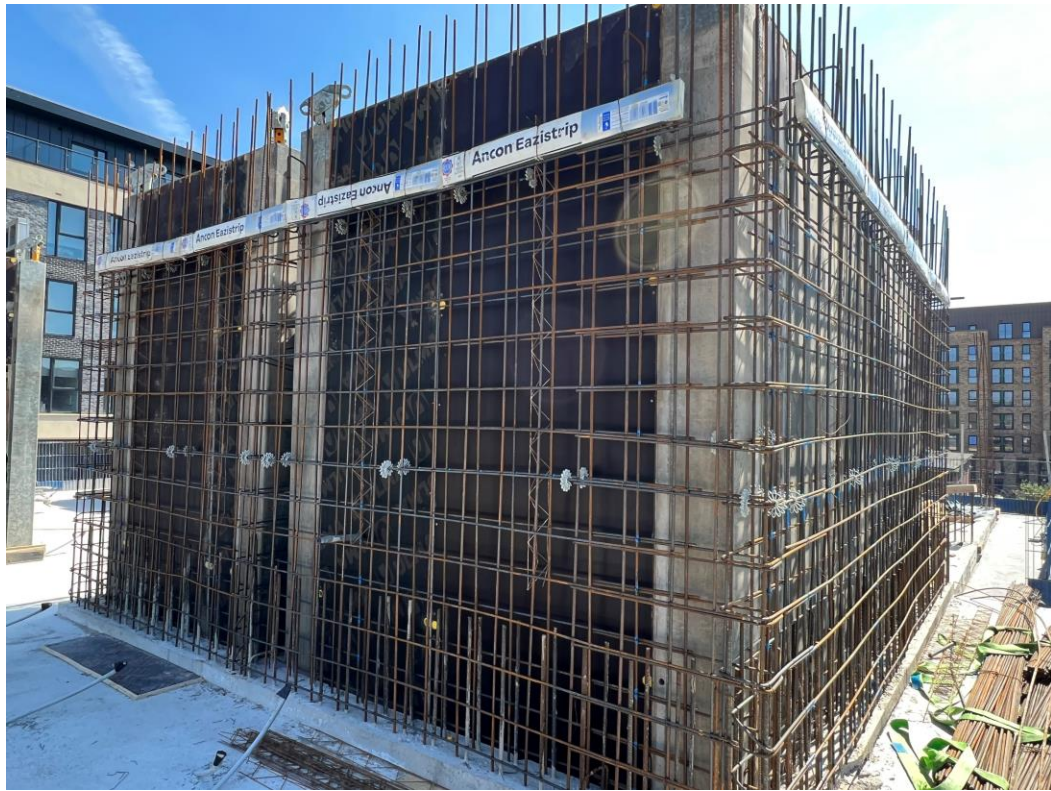
Block B lift and stair core structure
