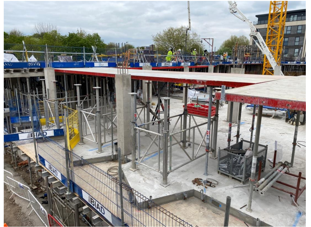
Block B PT floor slab preparation
