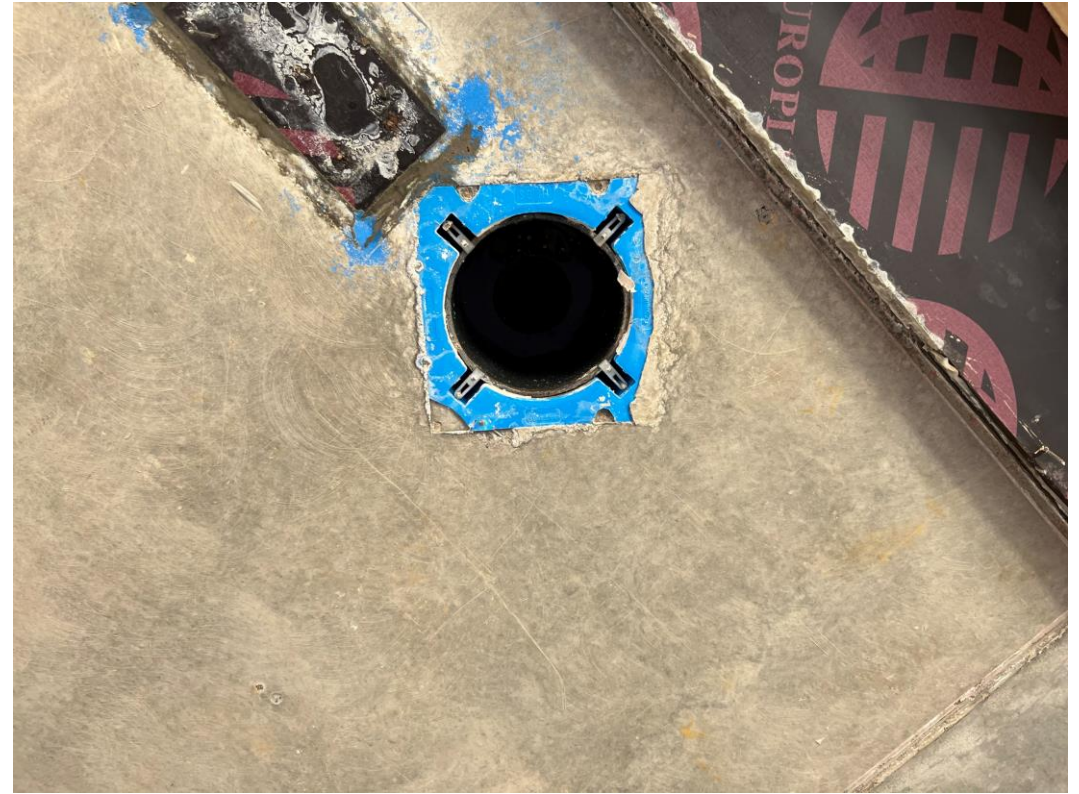
Fire collars installed
