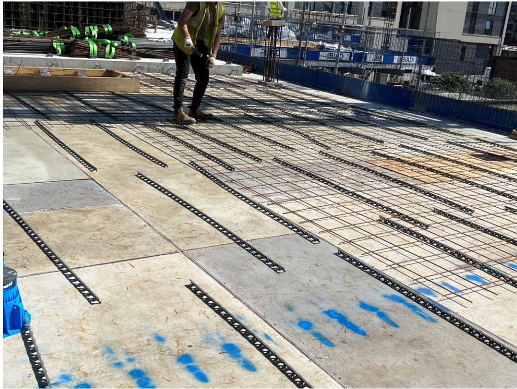
Block B PT floor slab preparation
