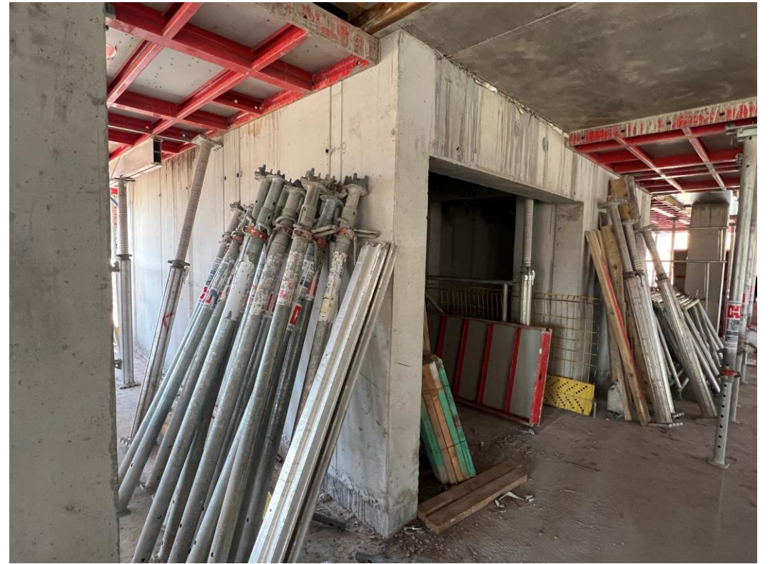
Block B lift and stair core structure
