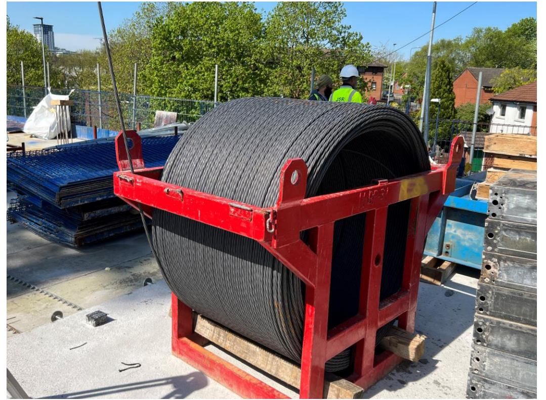
Block B PT floor slab preparation
