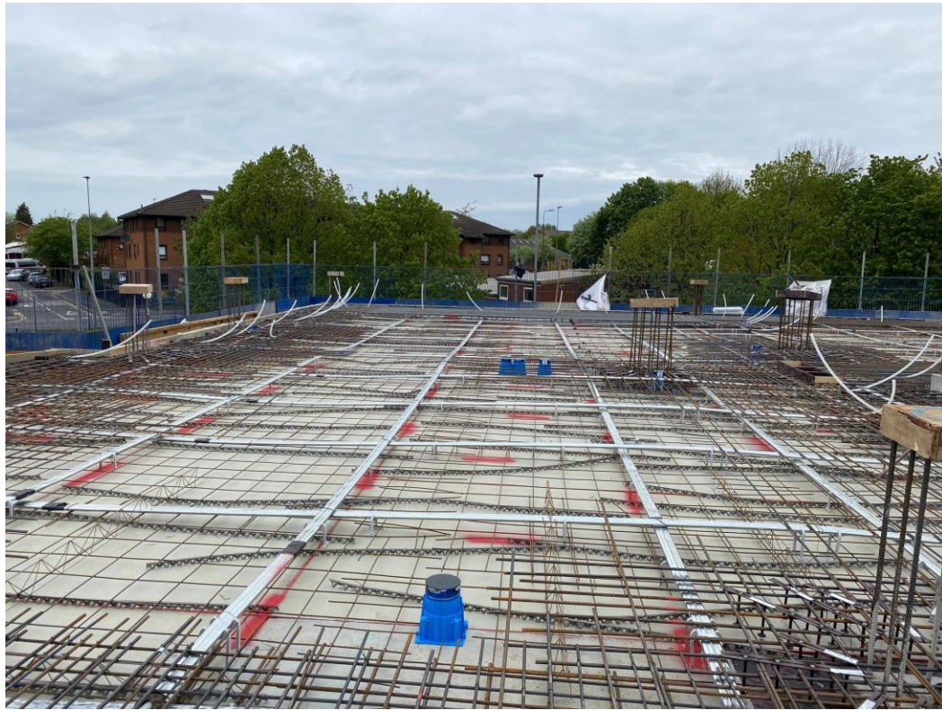
Block B PT floor slab preparation
