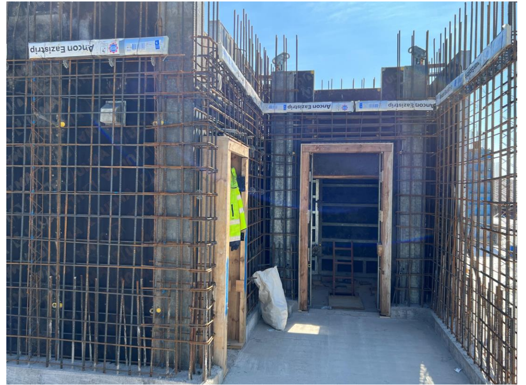
Block B lift and stair core structure
