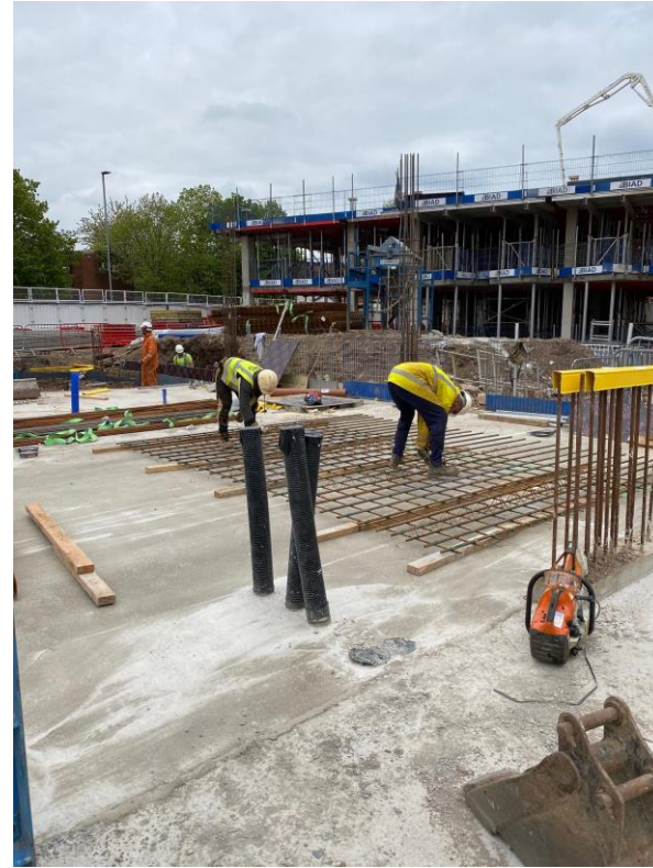
Block A slab poured
