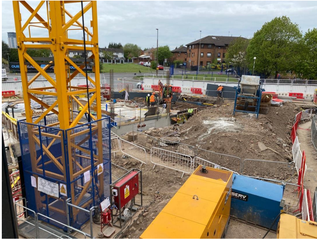
Block A site activity
