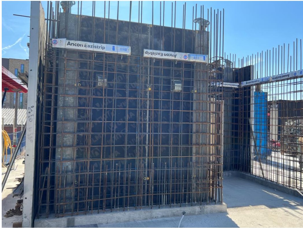
Block B lift and stair core structure
