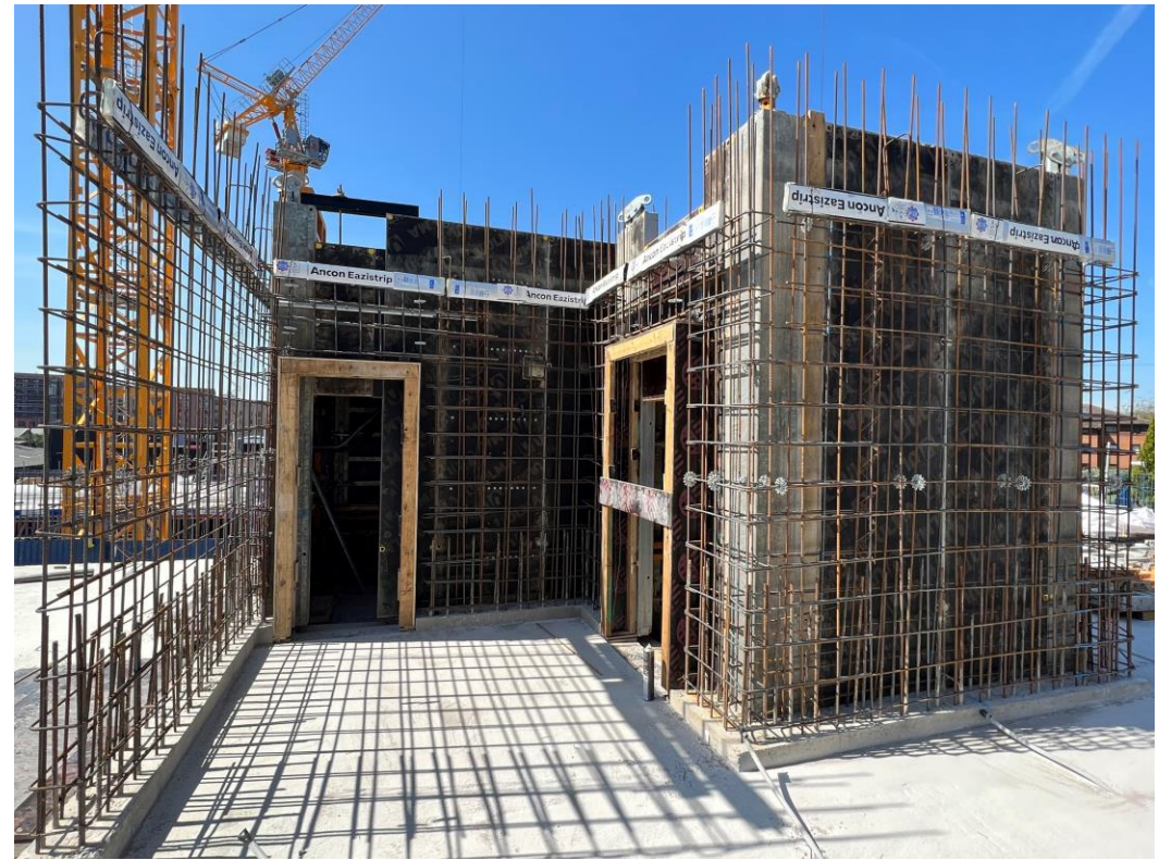
Block B lift and stair core structure
