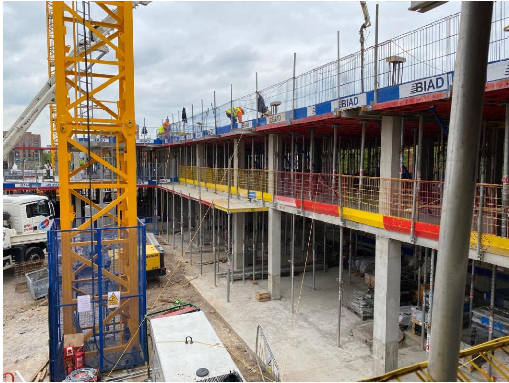
Block B superstructure
