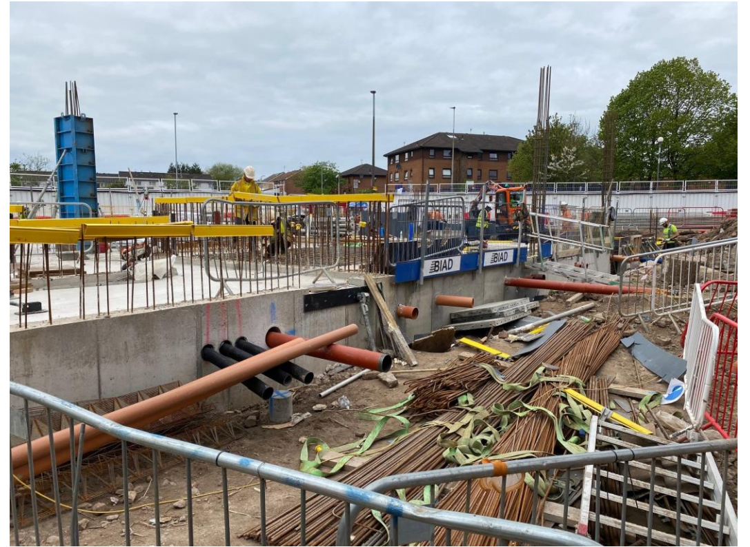
Block A substructure
