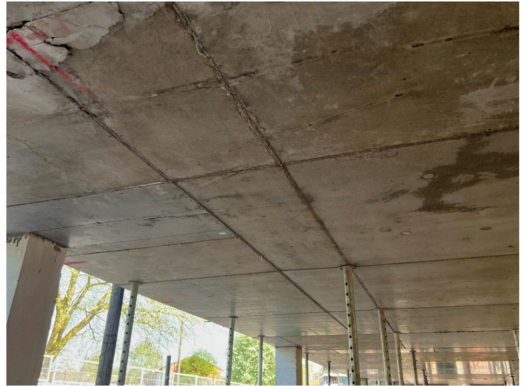
Block B first floor soffit
