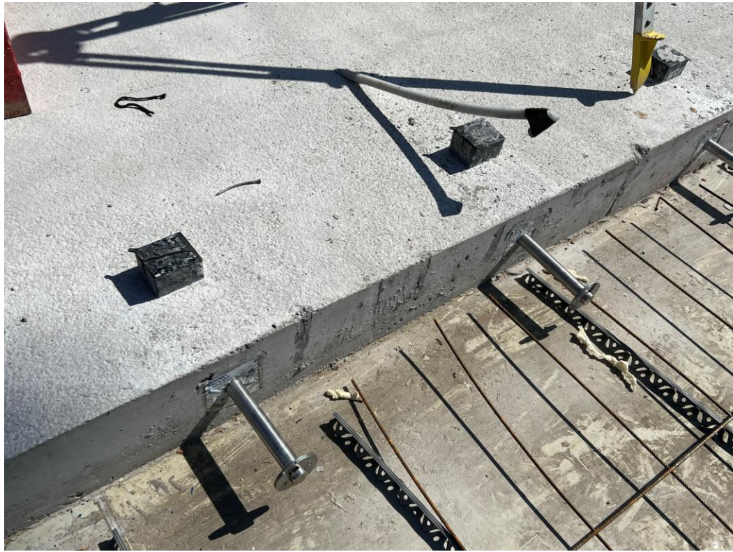
Block B PT floor slab preparation
