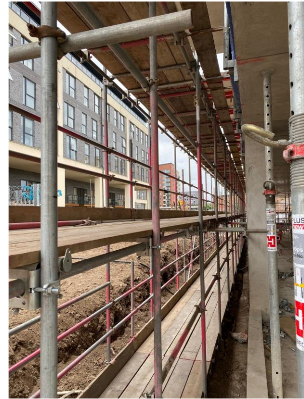
Block B scaffolding
