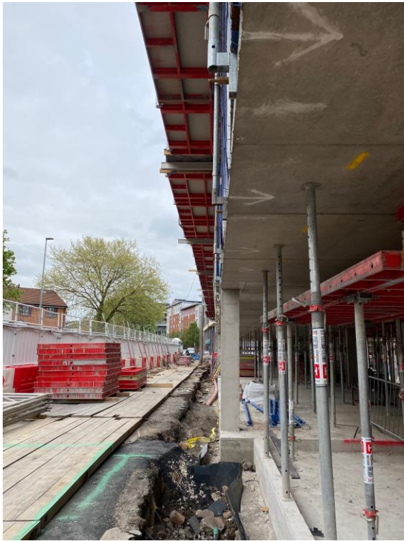
Block B superstructure
