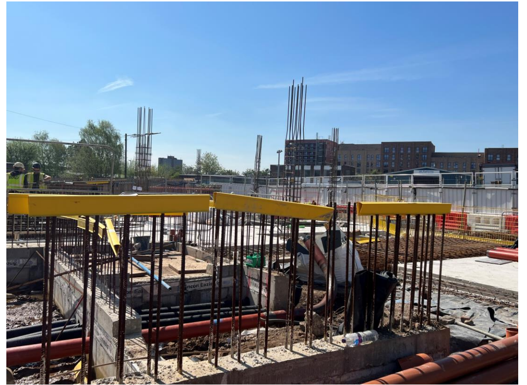
Block A substructure
