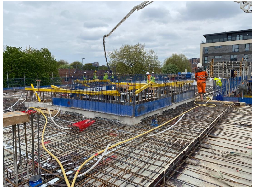
Block B PT floor slab preparation
