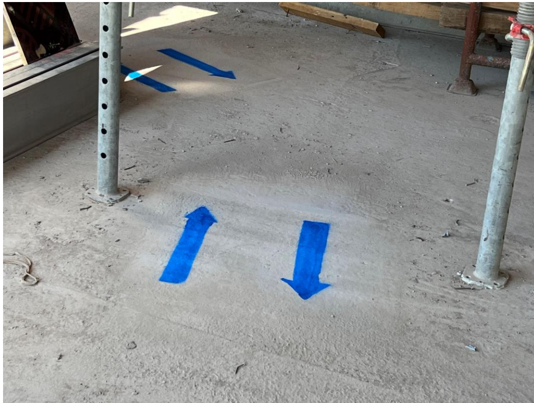
Site direction travel route
