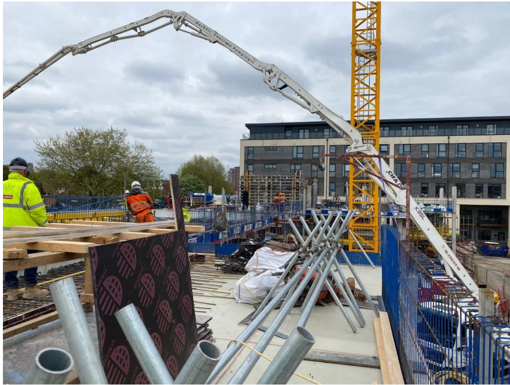
Block B PT floor slab preparation
