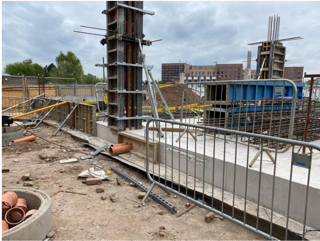
Block A column structure
