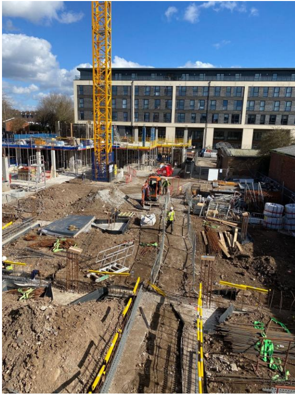
Block B concrete frame structure
