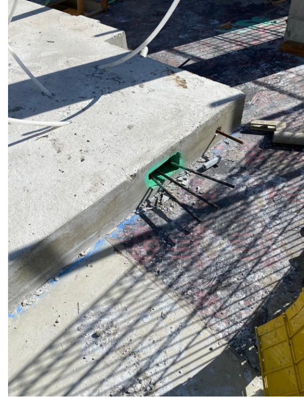
Block B first floor PT concrete slab structure
