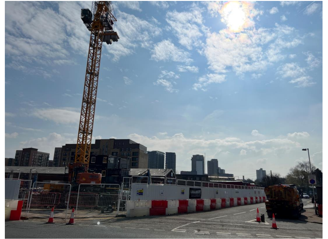
Ordsall Lane site view
