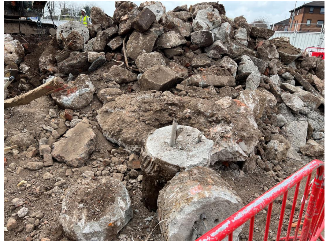
Block A pile cropping
