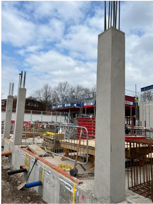
Block B concrete columns structure
