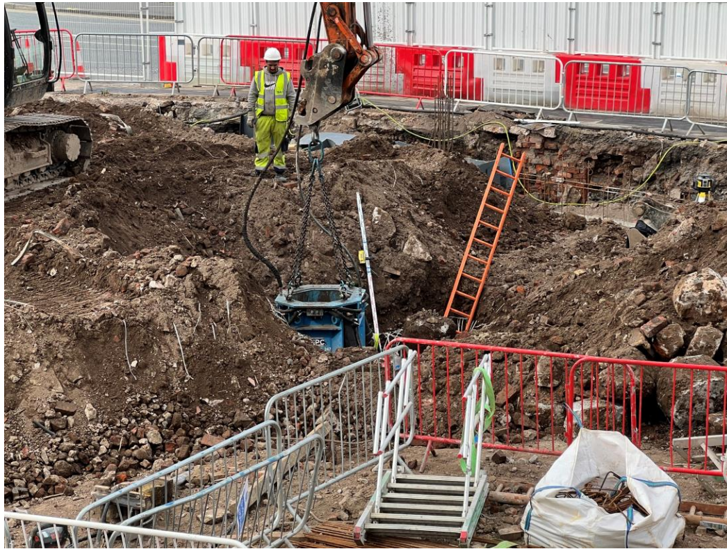
Block A pile cropping
