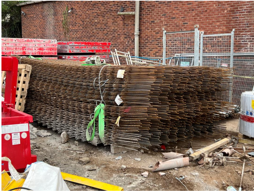
Floor slab reinforcement
