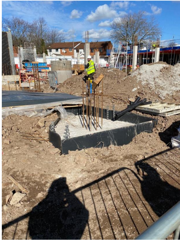
Reinforcement cages capping beams and columns
