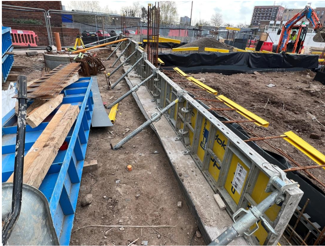
Block A floor slab, capping beams and columns
