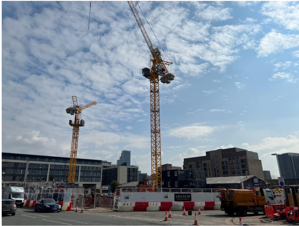
Ordsall Lane site view
