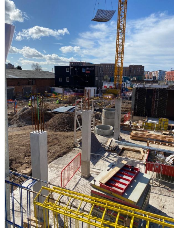
Block B concrete columns structure
