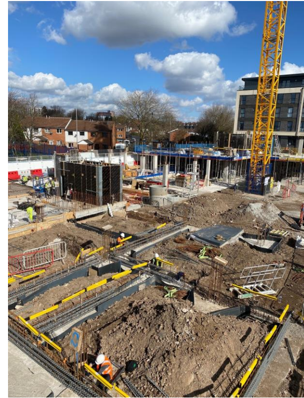
Block B concrete frame structure
