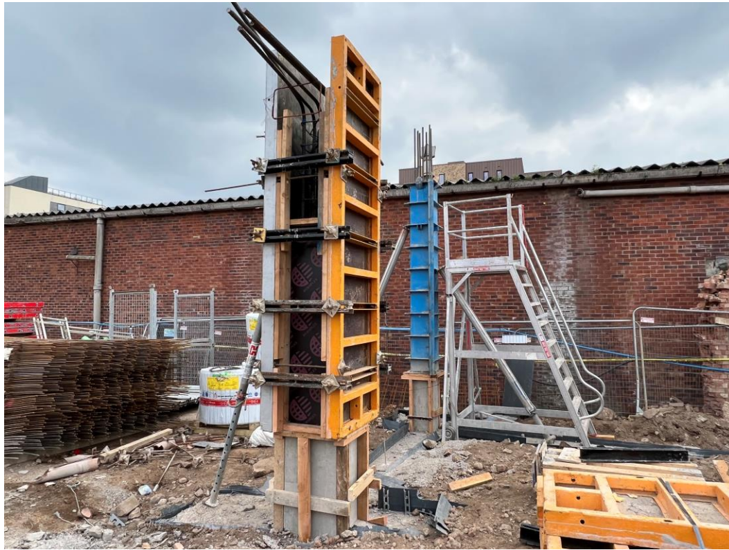
Block B concrete columns structure
