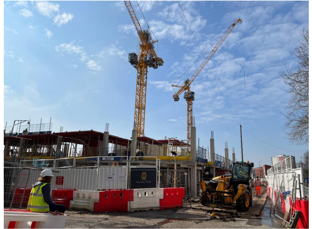
Ordsall Lane site view
