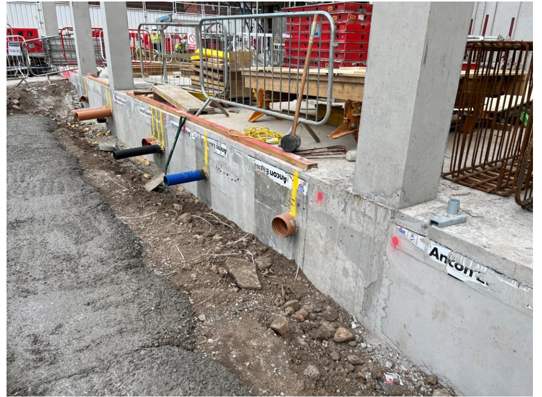
Block B concrete slab structure
