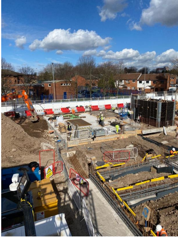
Block B concrete slab structure
