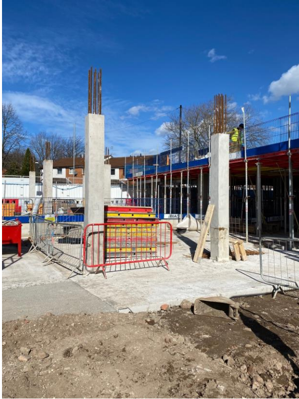
Block B concrete columns structure
