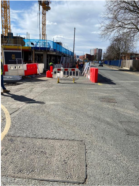
Ordsall Lane site view
