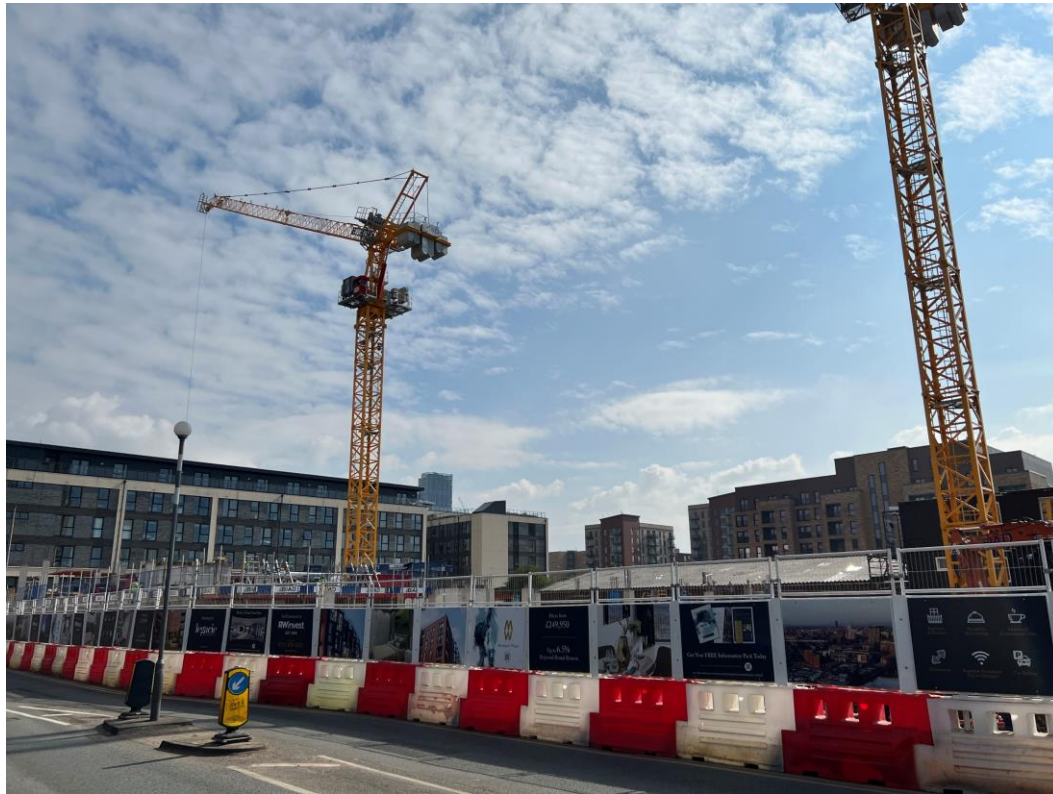
Ordsall Lane site view
