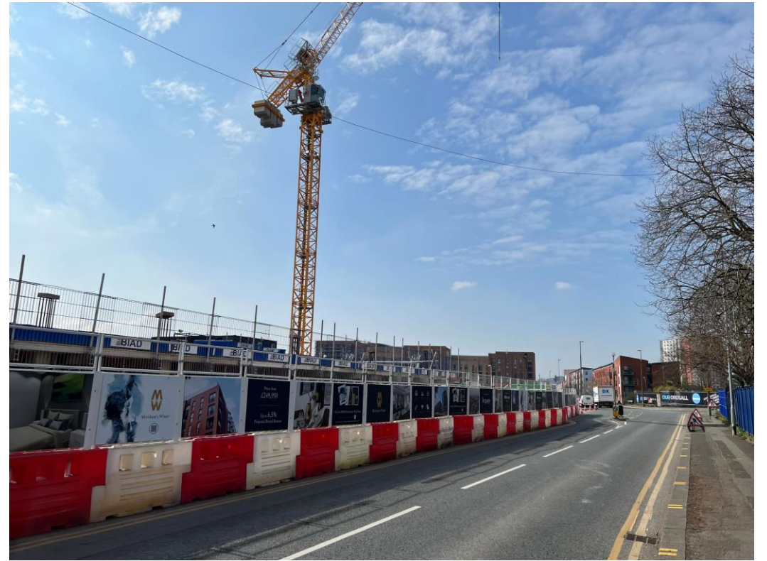
Ordsall Lane site view
