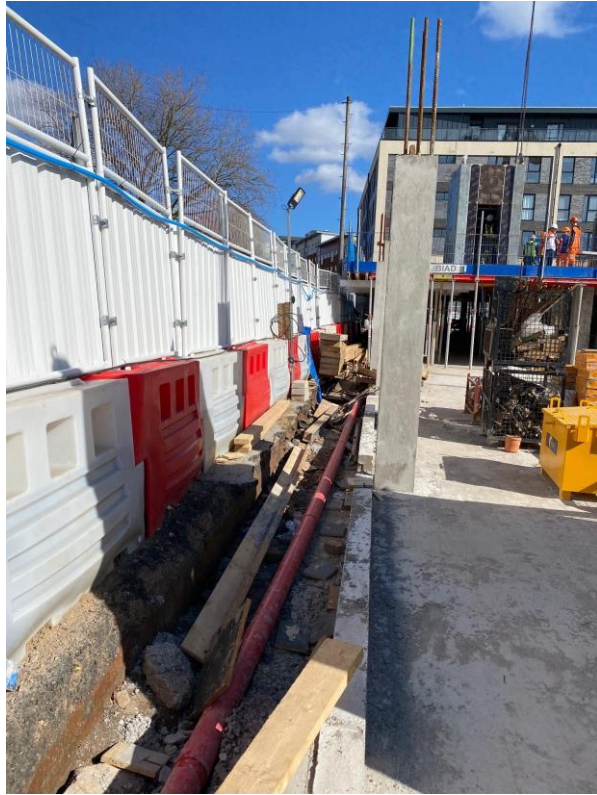
Ordsall Lane site view
