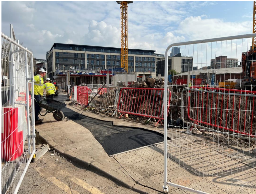
Ordsall Lane site view
