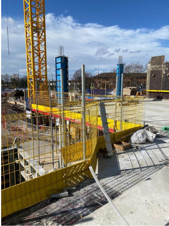
Block B first floor concrete slab & column structure
