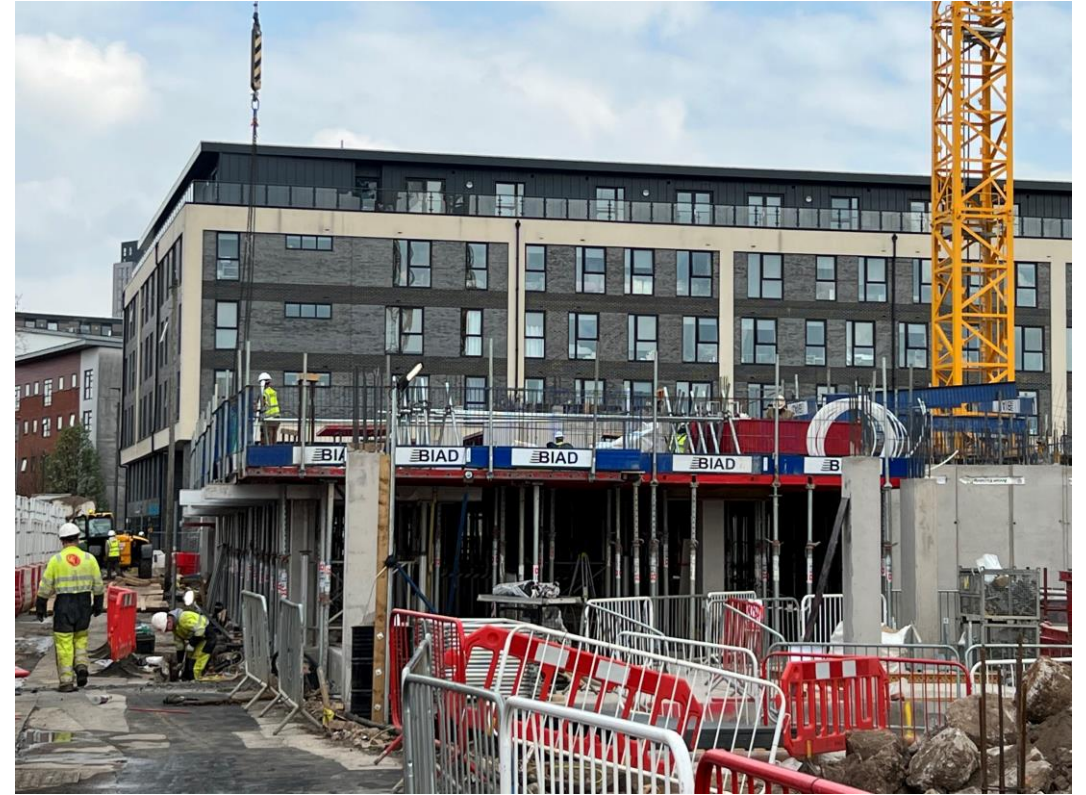
Ordsall Lane site view
