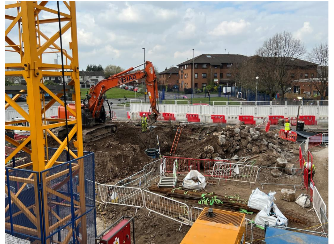
Block A pile cropping
