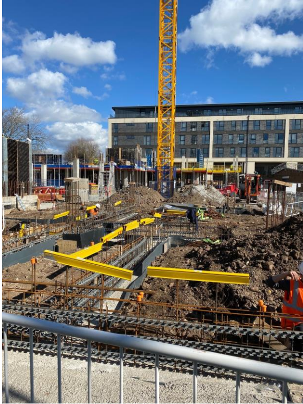
Reinforcement cages capping beams and columns
