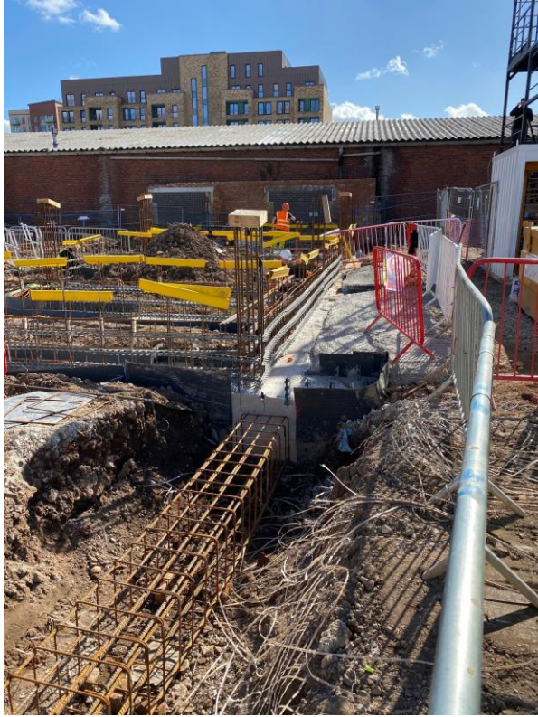
Reinforcement cages capping beams and columns
