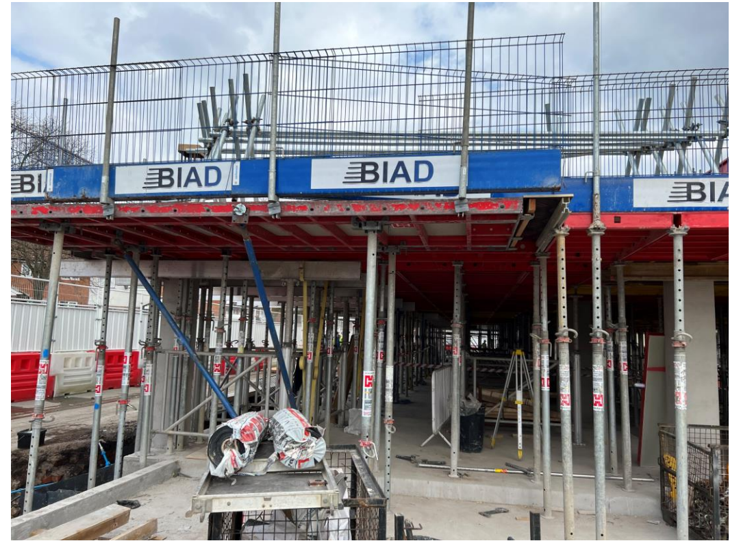
Block B First floor concrete PT slab structure
