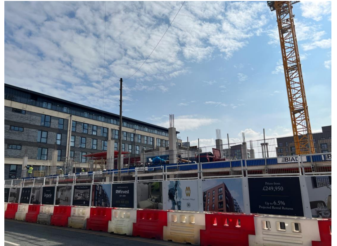
Ordsall Lane site view
