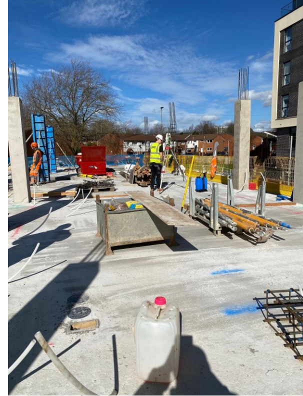
Block B first floor concrete slab & column structure
