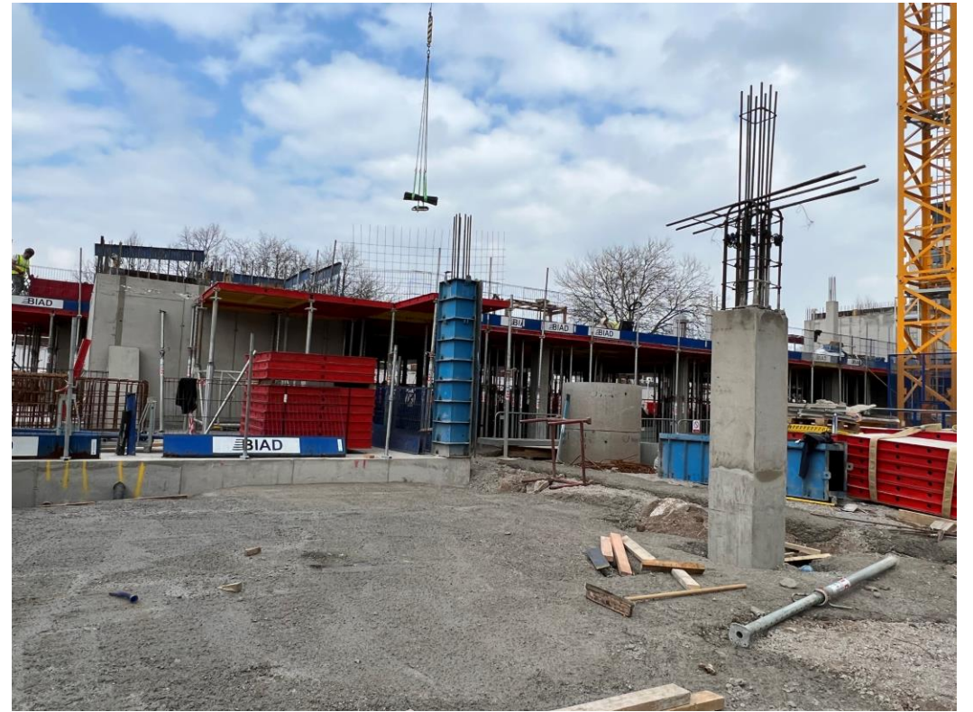
Block B concrete columns structure
