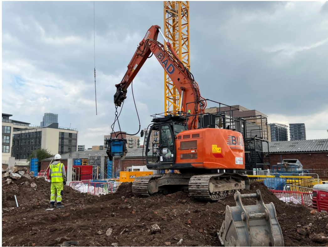
Block A pile cropping
