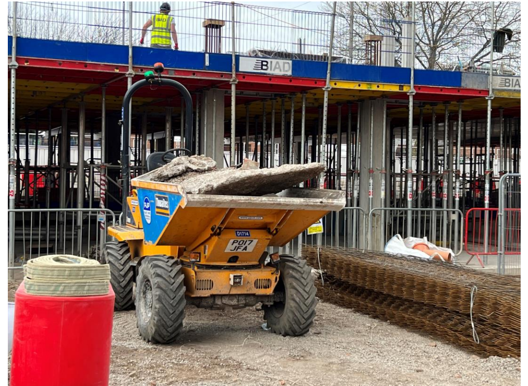
Site plant and machinery
