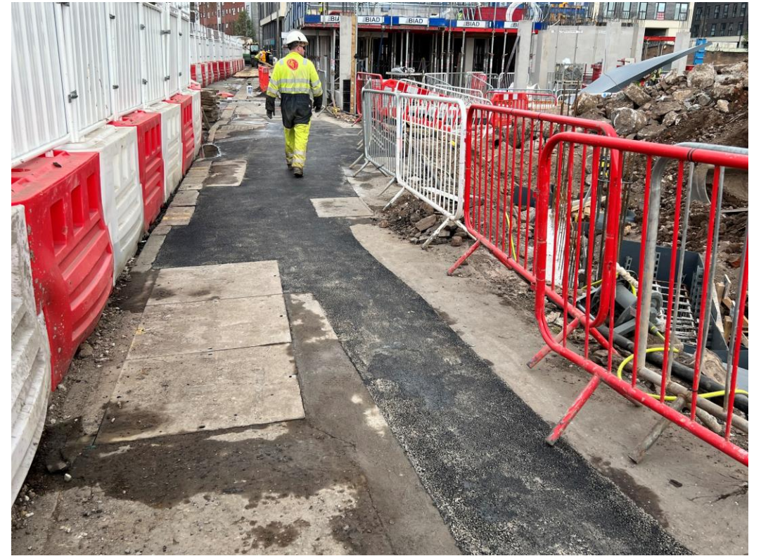
Ordsall Lane site view
