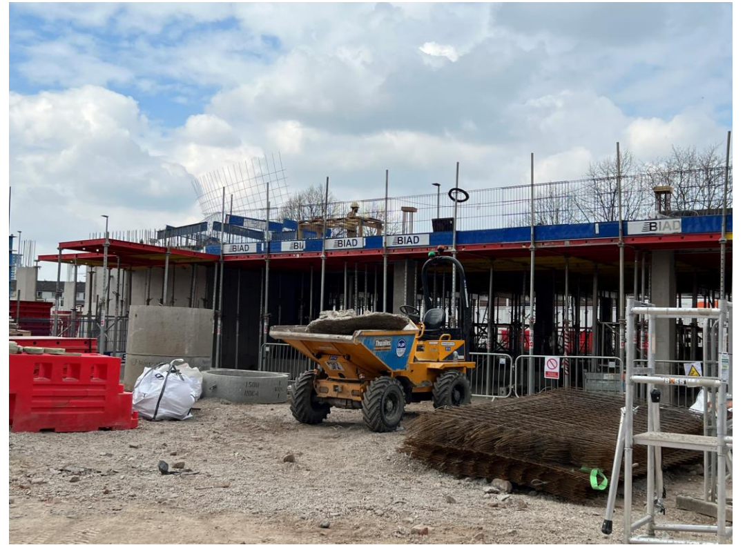
Site plant and machinery
