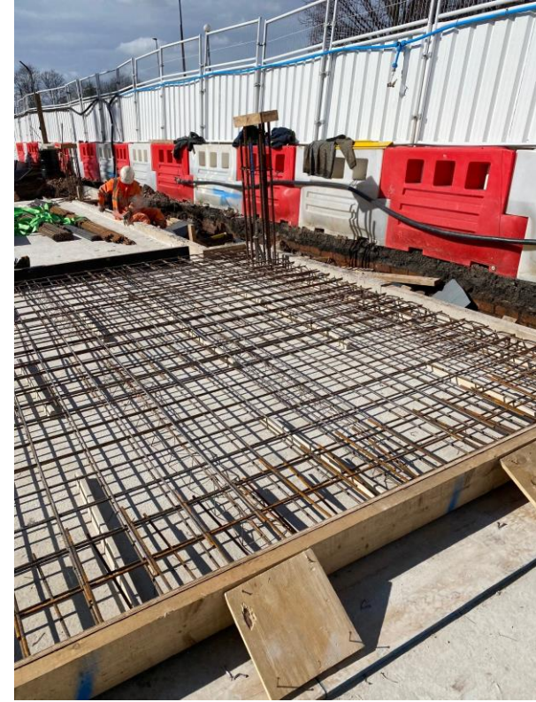
Block B concrete slab structure
