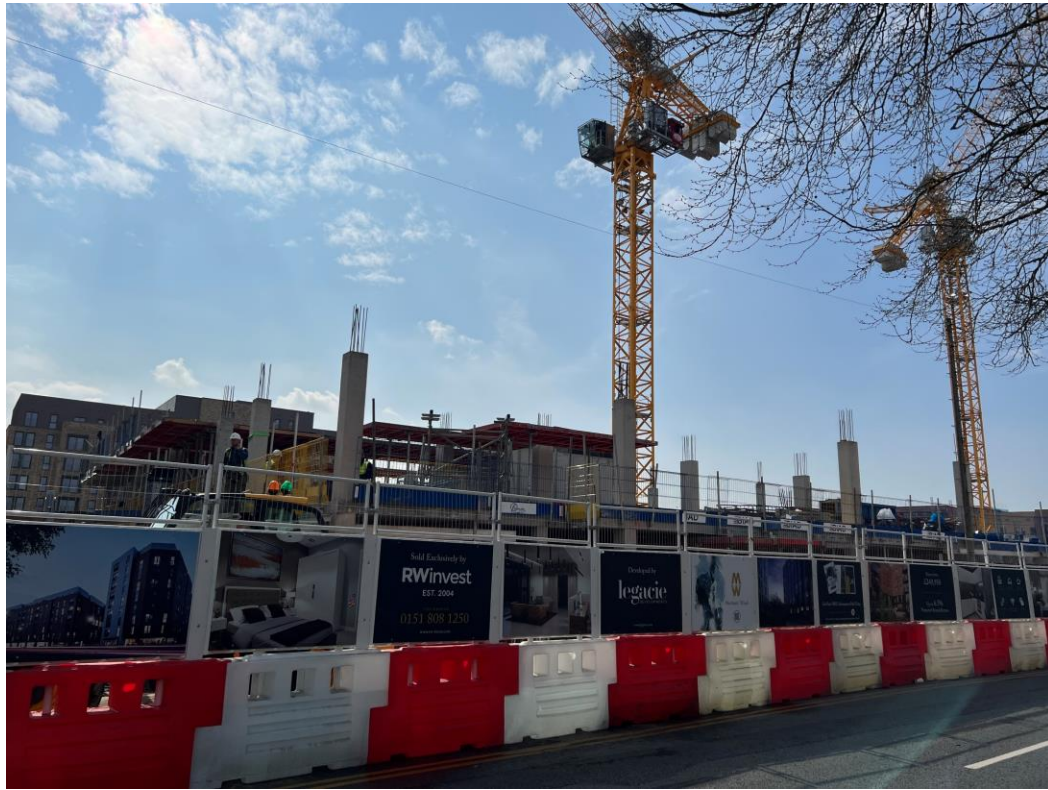
Ordsall Lane site view
