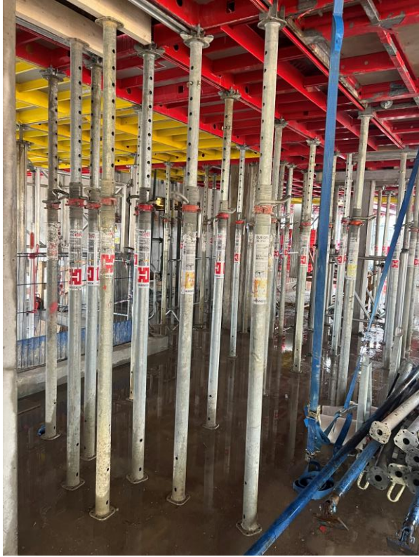
Block B concrete framework shuttering
