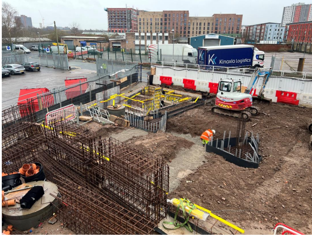
Block A pad foundation under construction
