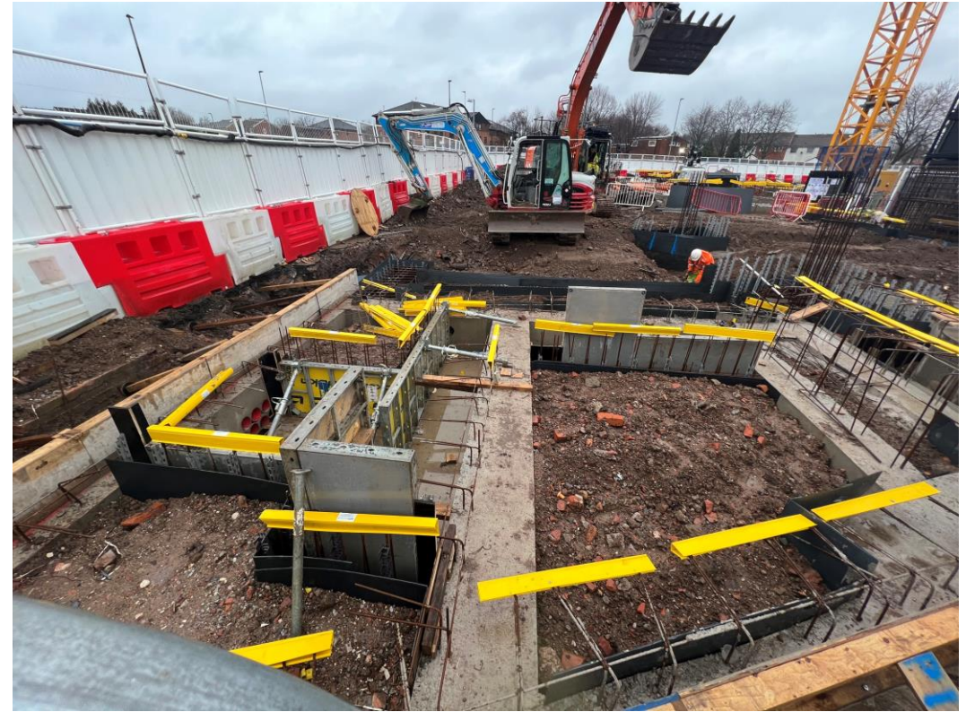
Sub-station capping beam concrete foundations
