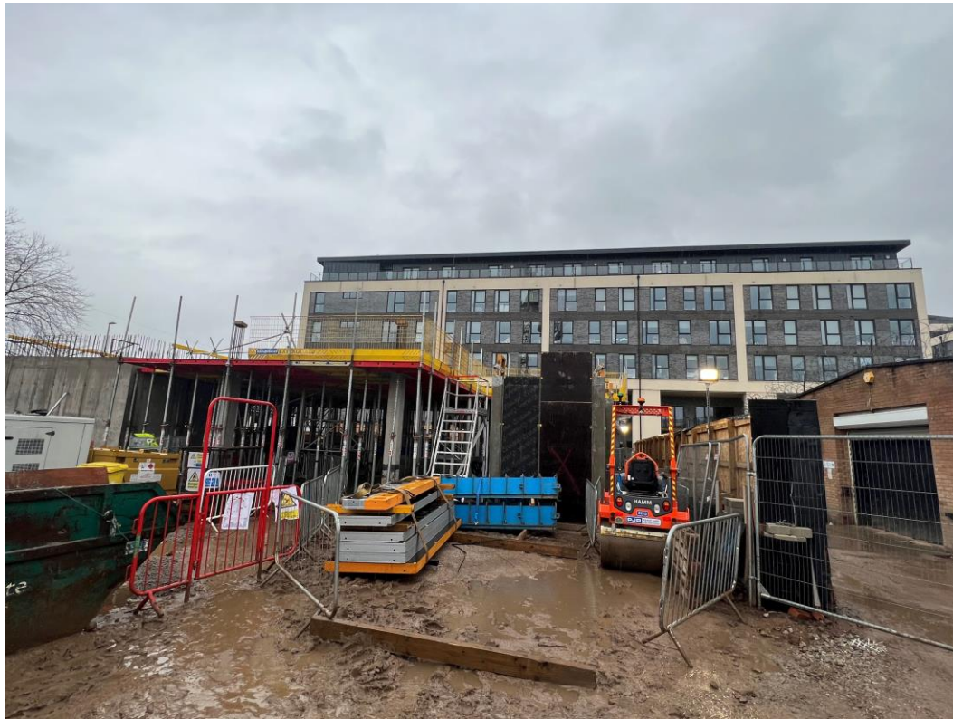
Block B concrete framework and upper floor slab construction
