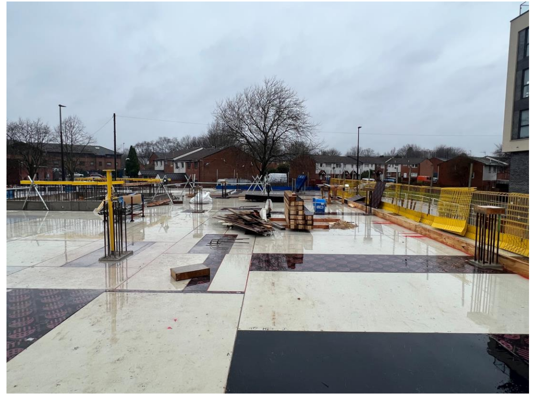
Block B concrete framework shuttering
