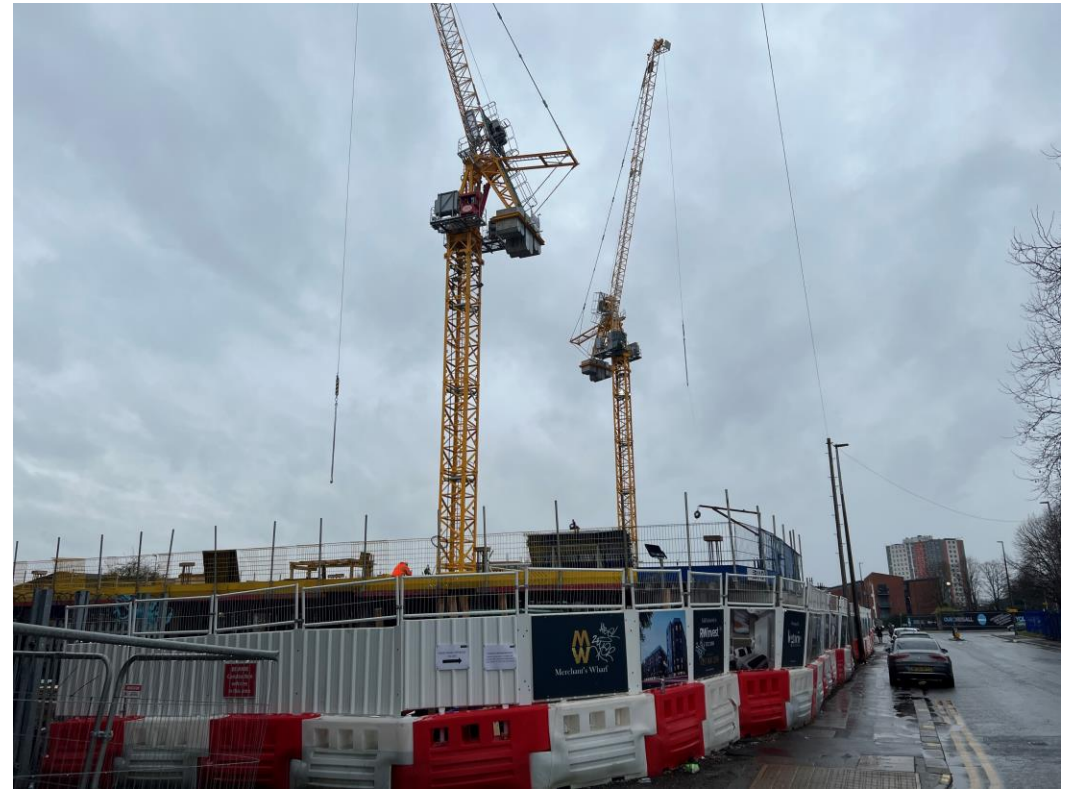
Ordsall Lane site view
