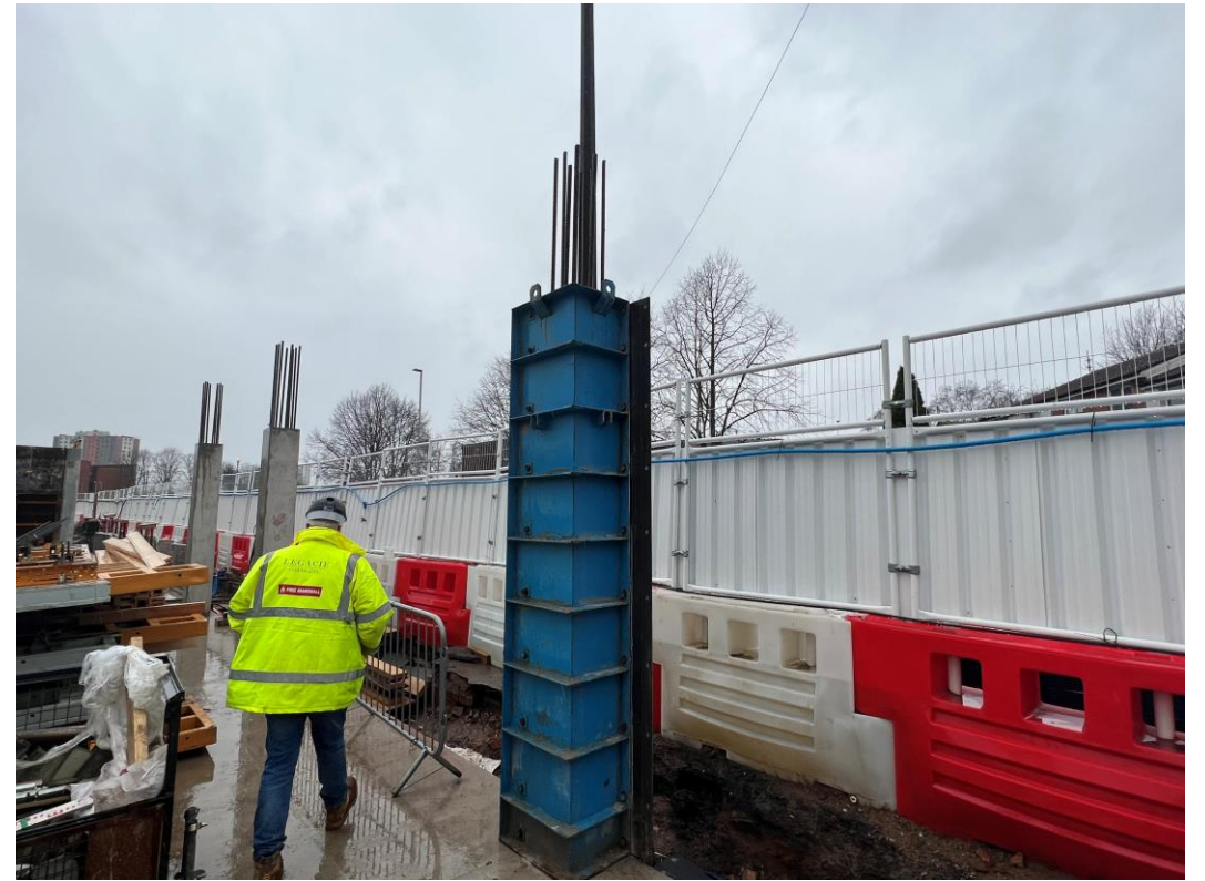
Block B floor slab installed & column construction
