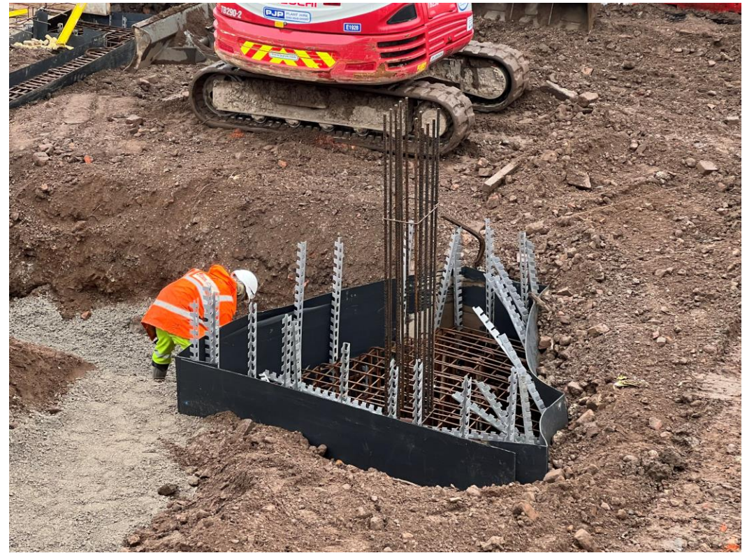
Block A pad foundation under construction
