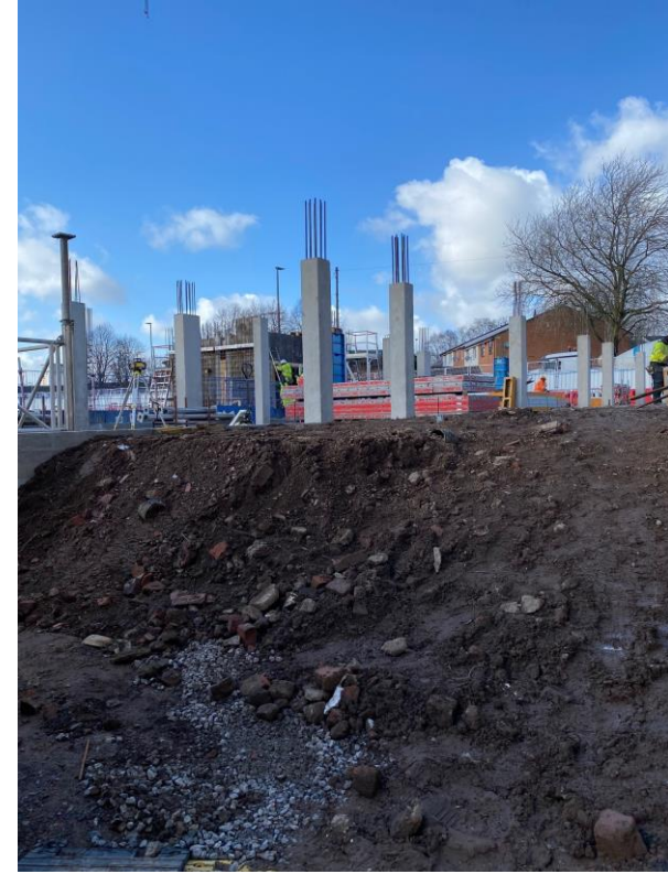
Concrete column structure
