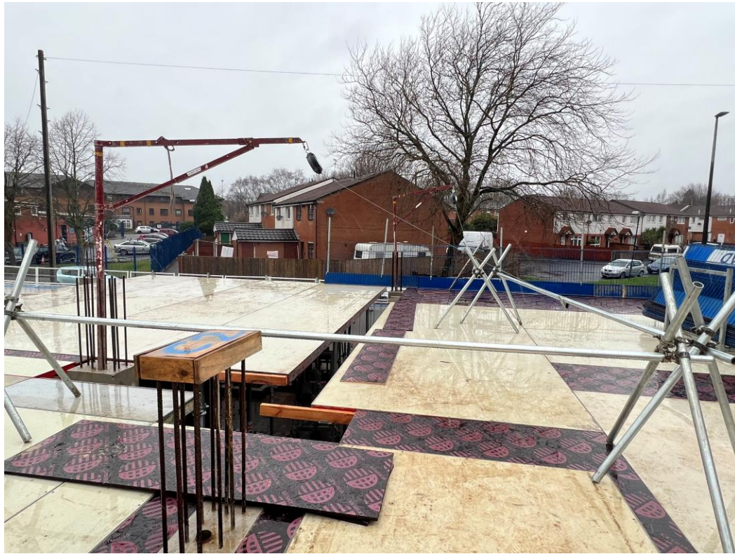
Block B concrete framework shuttering
