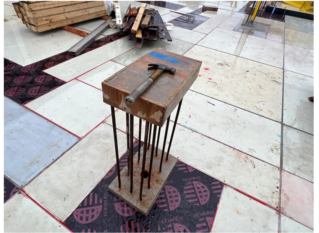
Block B concrete framework shuttering
