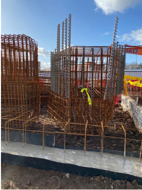
Reinforcement cages stored pad foundations
