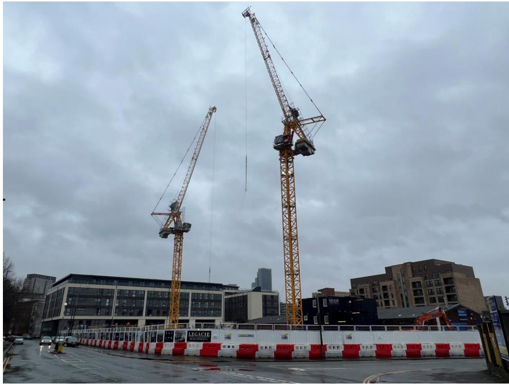
Ordsall Lane site view
