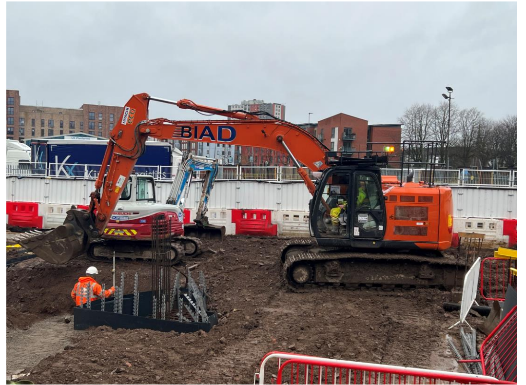
Block A general site activity
