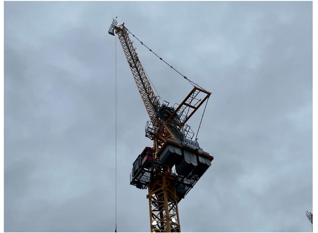
Cranes in use
