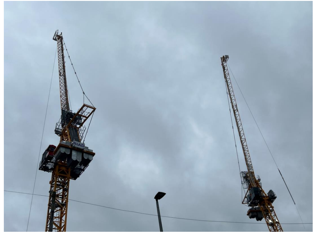
Ordsall Lane site view
