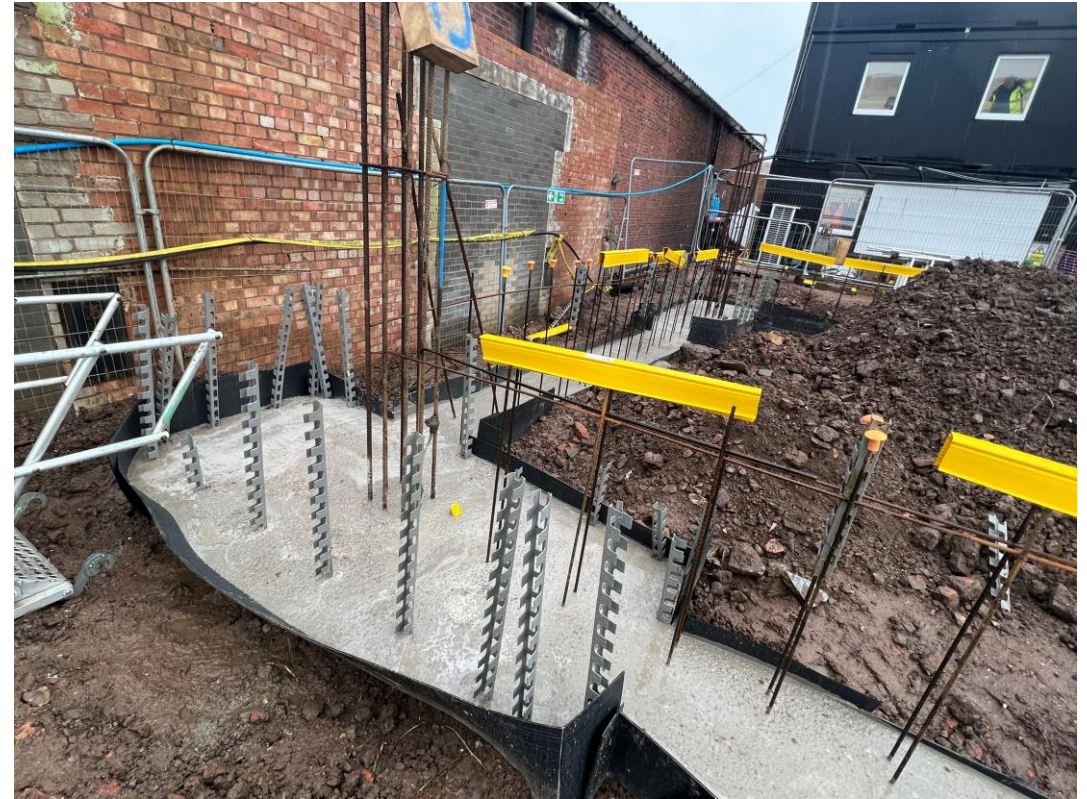
Block B capping beam under construction
