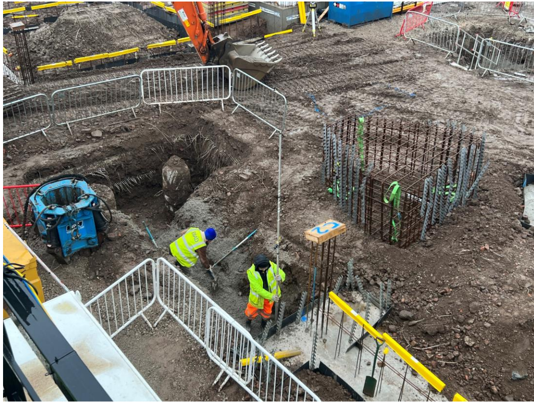
Block B pile cropping
