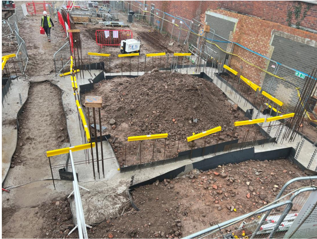
Block B capping beam under construction
