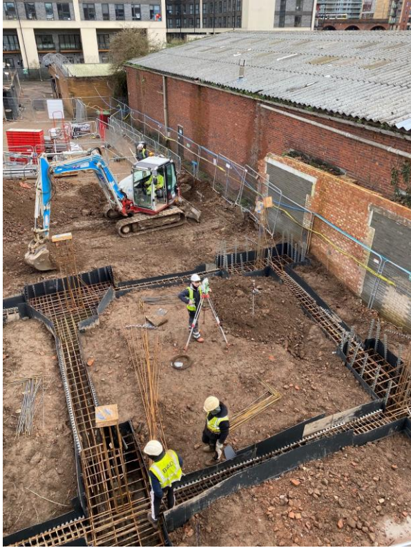
Block B capping beam under construction
