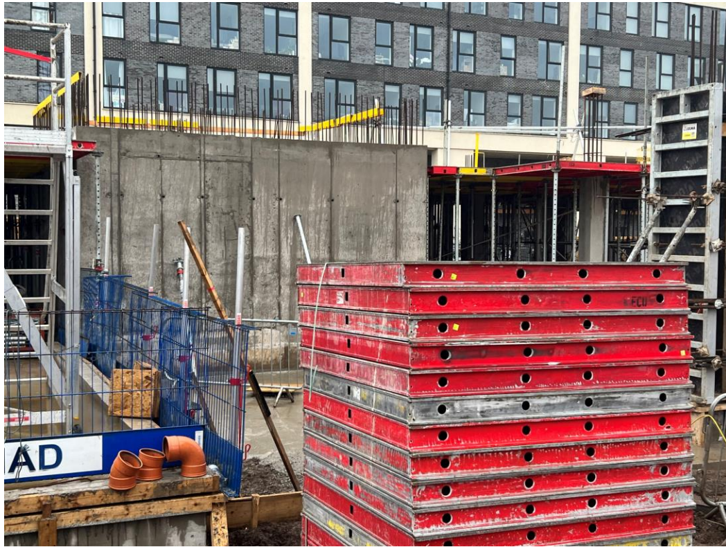
Block B stair core construction
