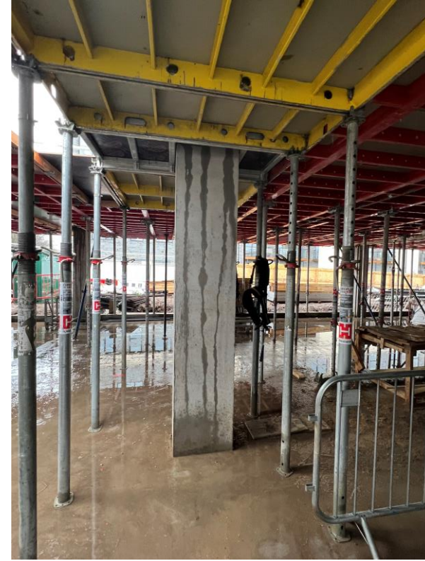
Block B concrete framework shuttering
