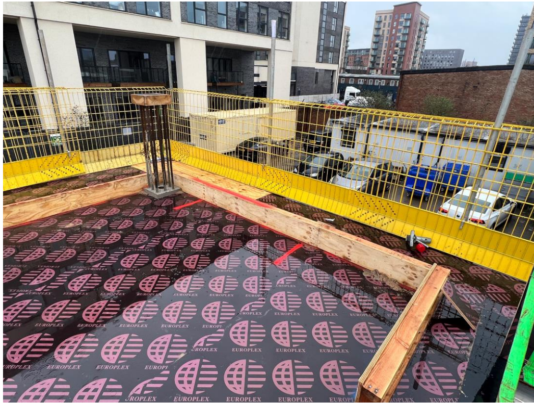
Block B concrete framework shuttering
