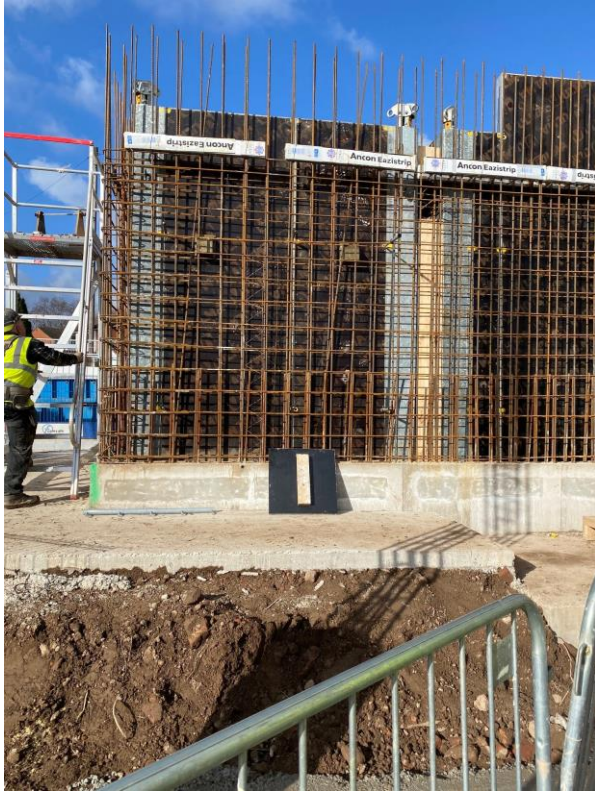
Block B stair core under construction
