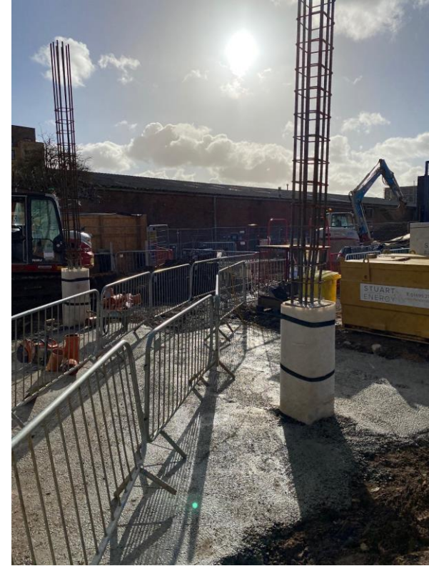
Concrete column structure
