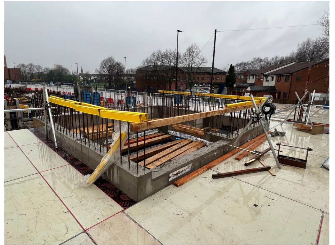
Block B concrete framework shuttering
