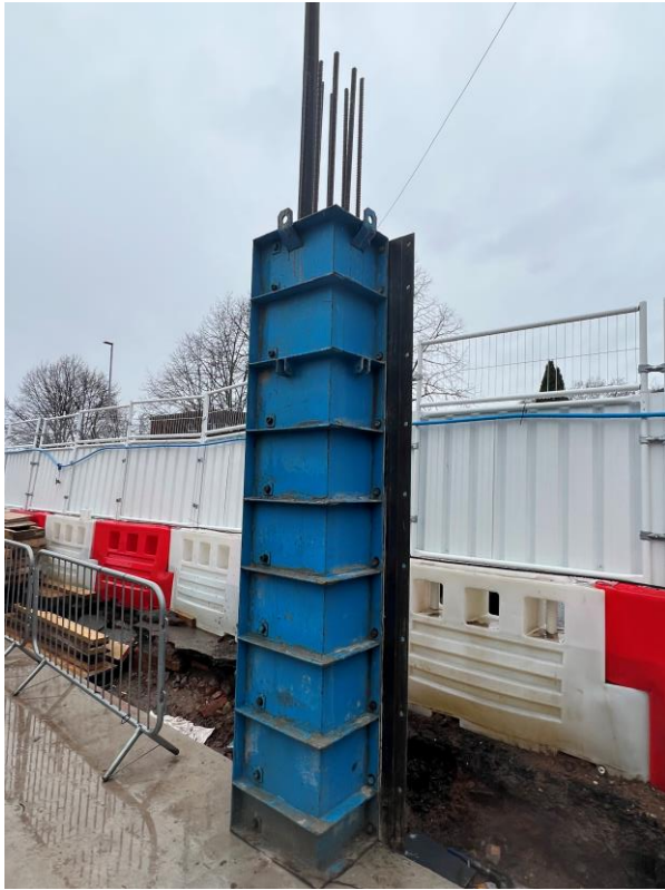
Block B floor slab installed & column construction
