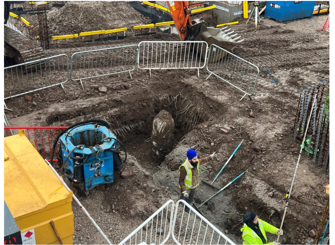
Block B pile cropping
