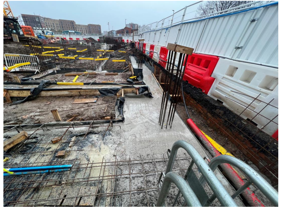
Block B capping beams installed
