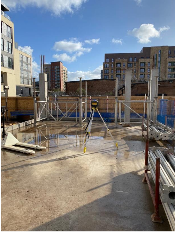
Concrete column structure
