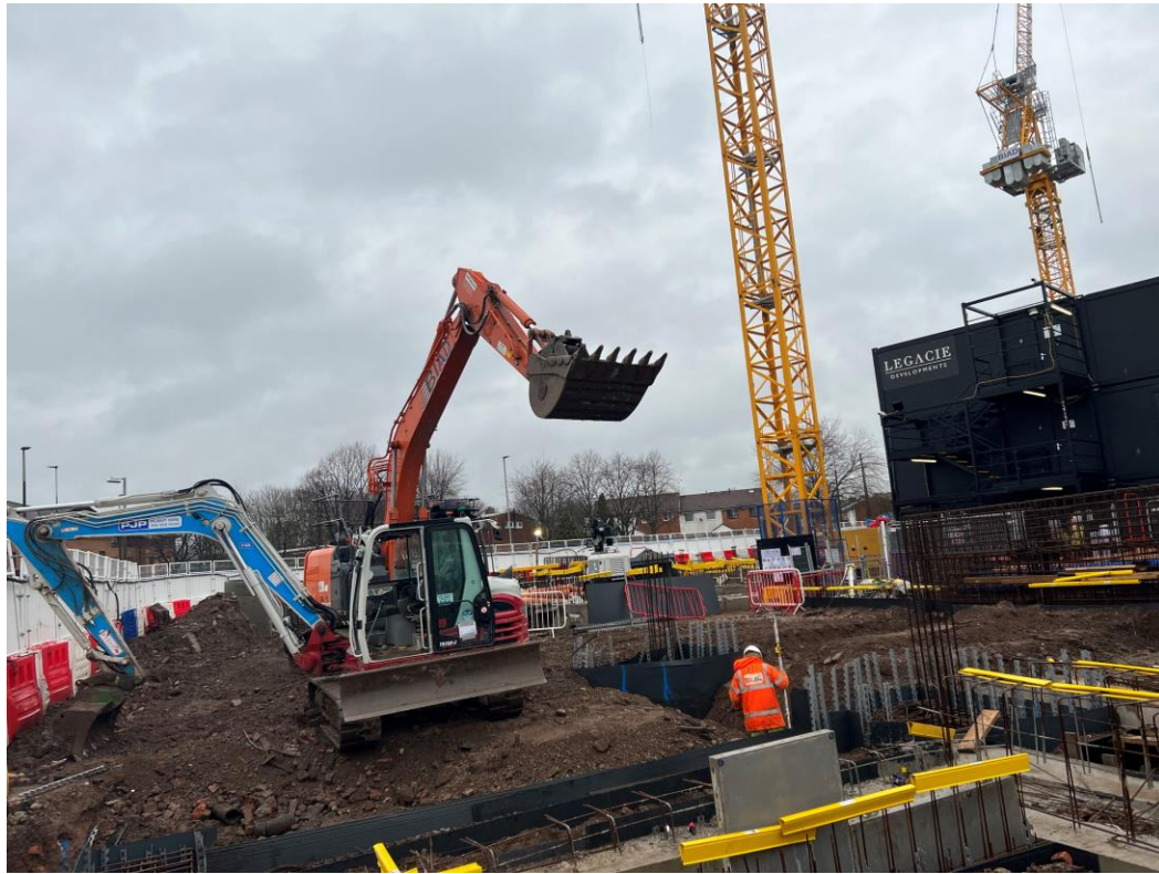
Block A general site activity
