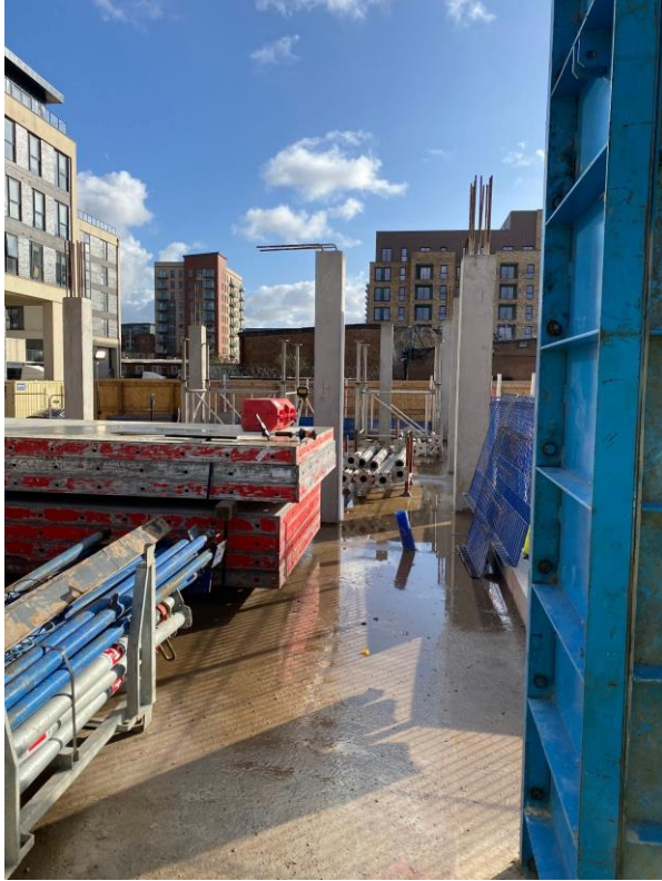
Concrete column structure
