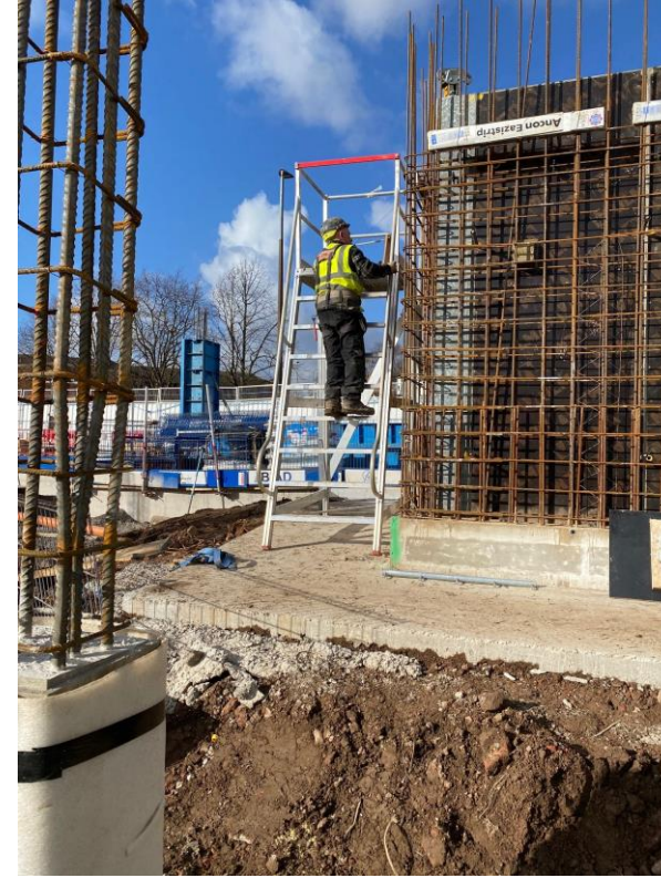
Block B stair core under construction
