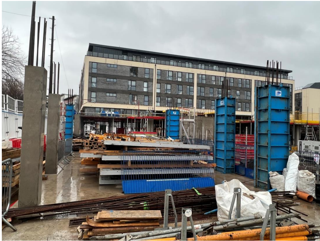
Block B floor slab installed & column construction
