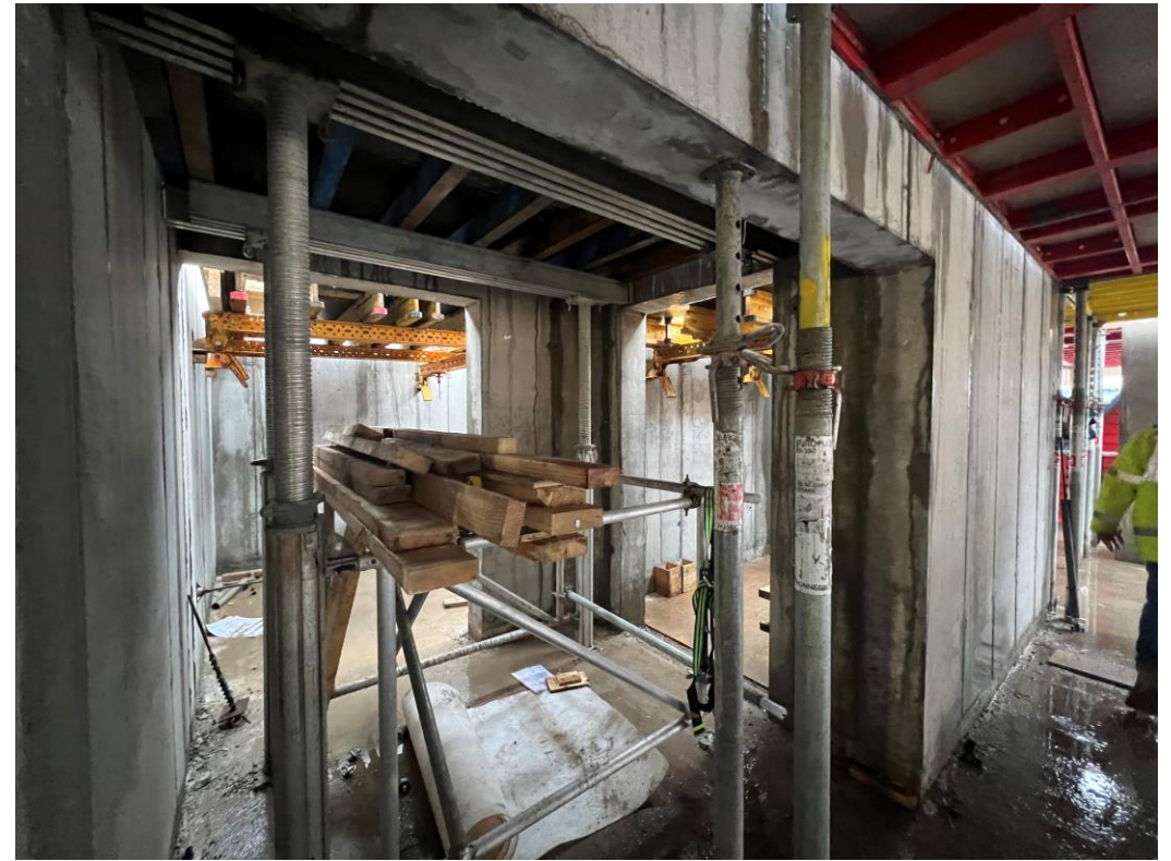
Block B stair core construction
