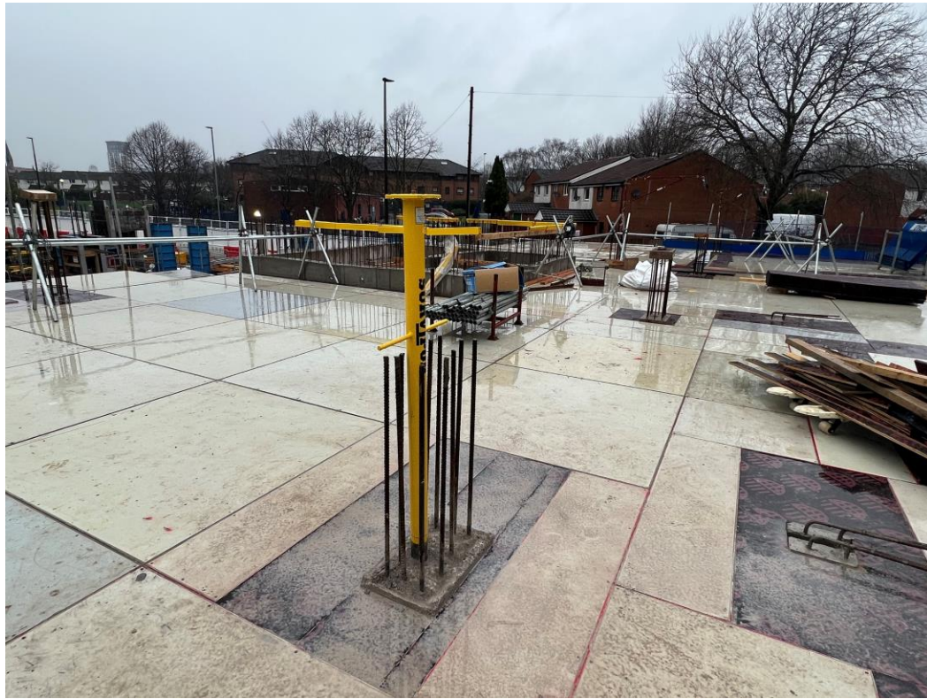
Block B concrete framework shuttering
