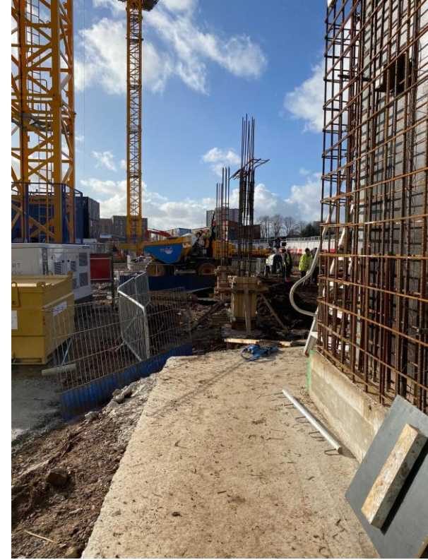
Block B stair core under construction
