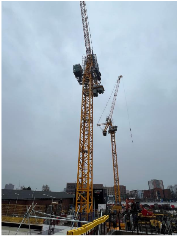
Cranes in use
