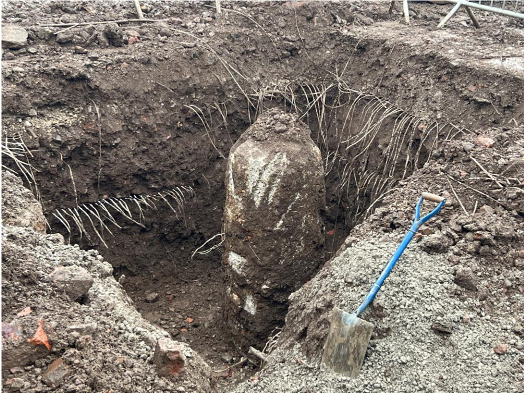
Block B pile cropping
