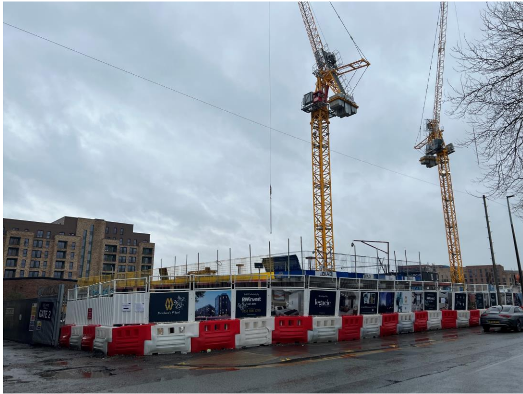
Ordsall Lane site view
