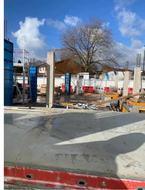
Concrete column structure
