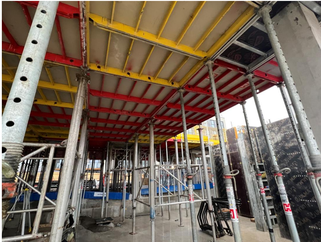
Block B concrete framework shuttering
