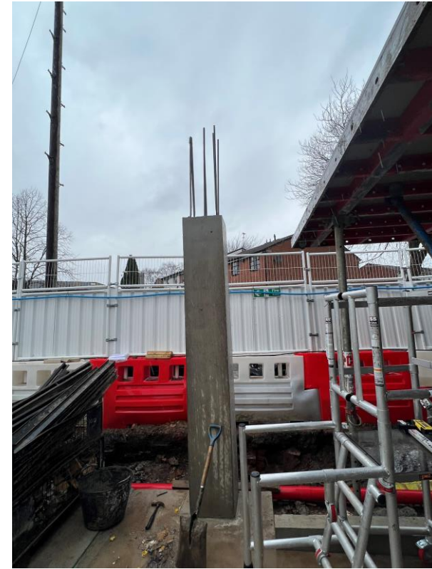
Block B floor slab installed & column construction
