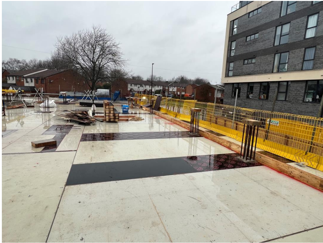
Block B concrete framework shuttering
