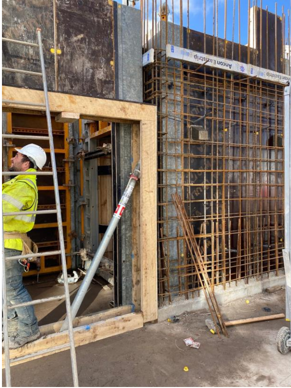
Block B stair core under construction
