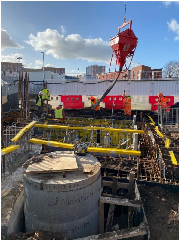
Sub-station capping beam concrete foundations poured
