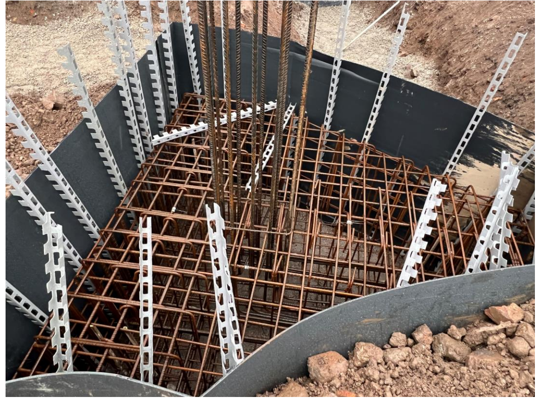
Block B pad foundation construction
