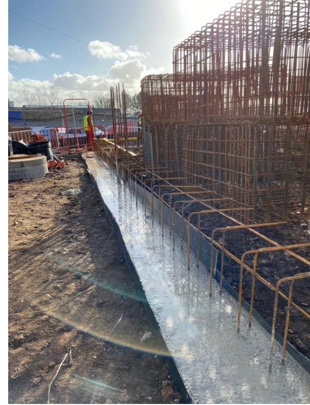
Capping beam concrete poured
