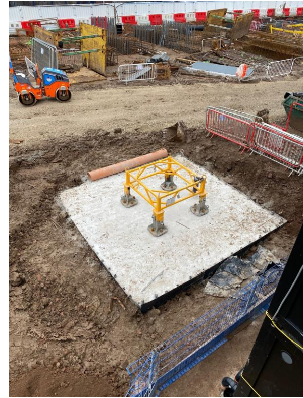
Lift core cast
