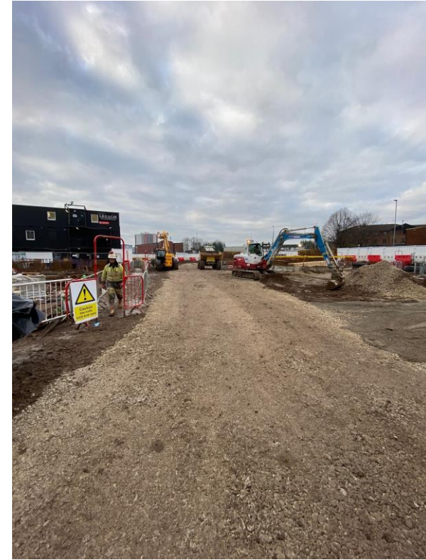
Site activity plant & machinery
