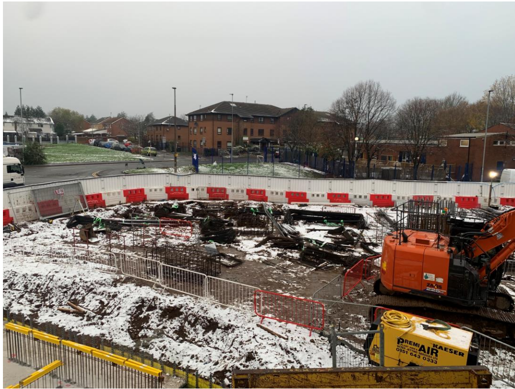
Foundation reinforcement cages being formed and stored
