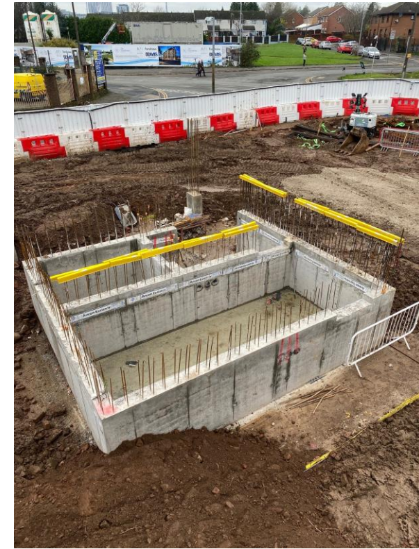
Core substructure installed
