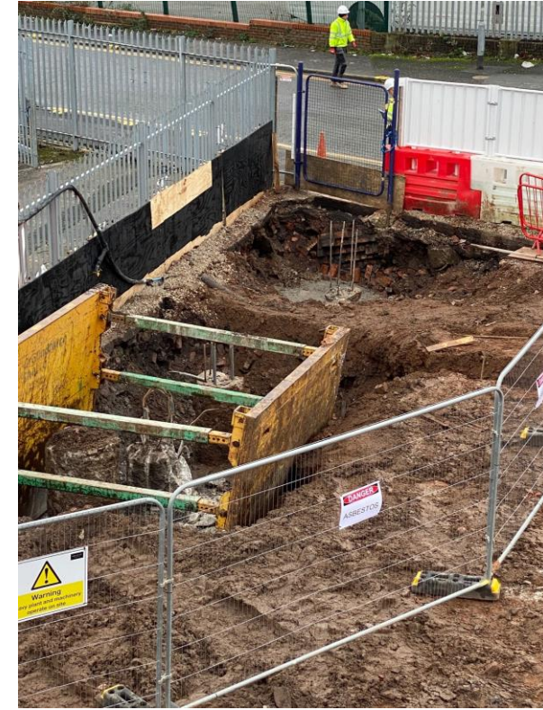
Block B – Temporary retaining structure onsite
