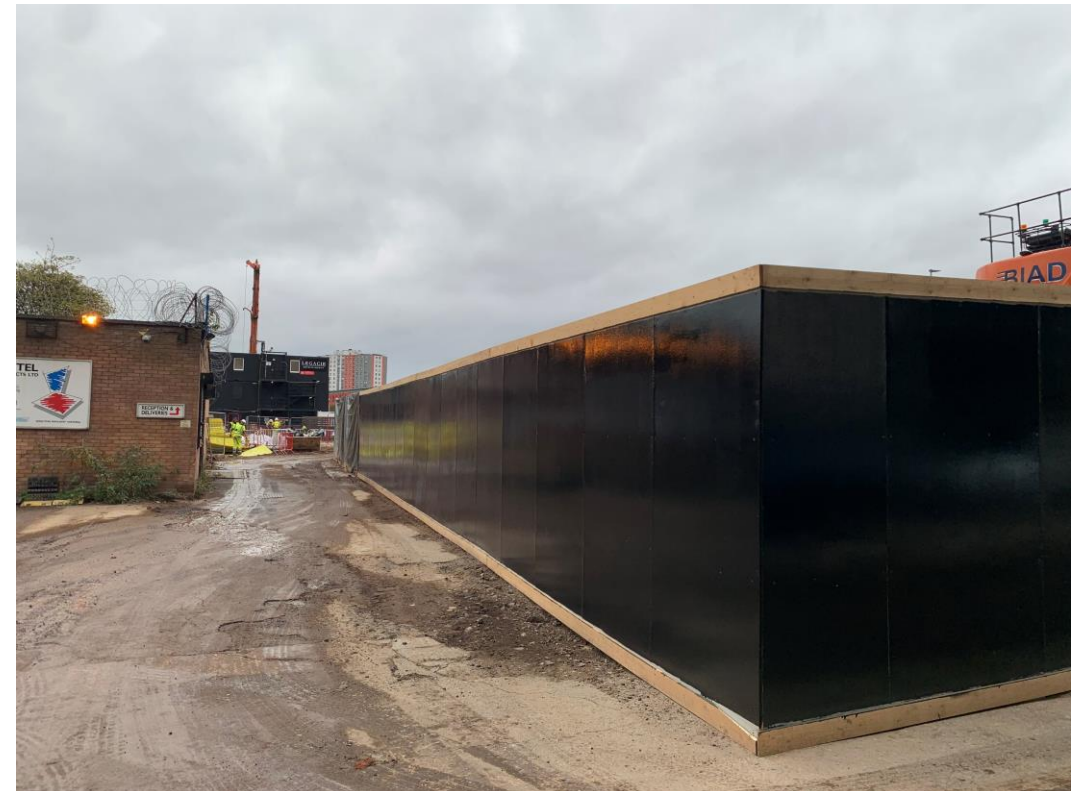
Worral Lane site plant & deliveries entrance
