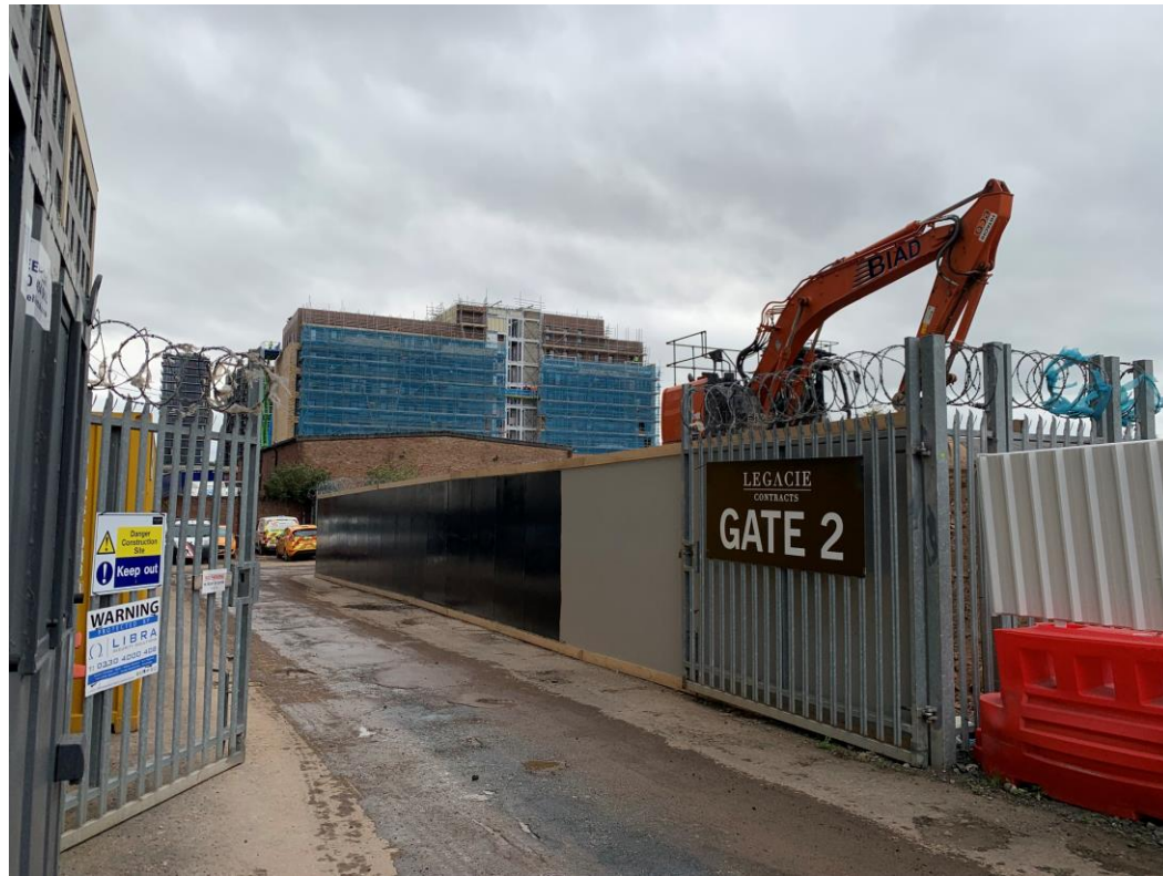
Dyer Street site plant & deliveries entrance
