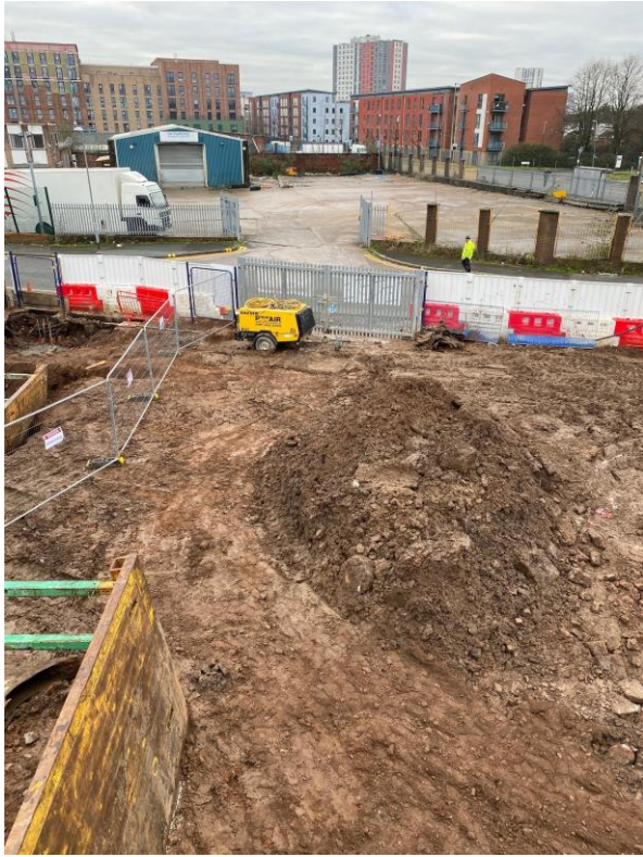
Site hoardings in place
