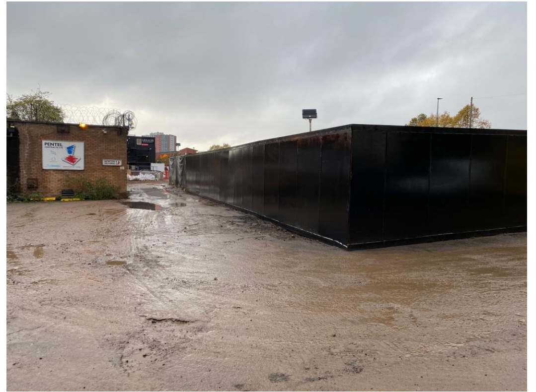
Worrall Lane site plant & deliveries entrance
