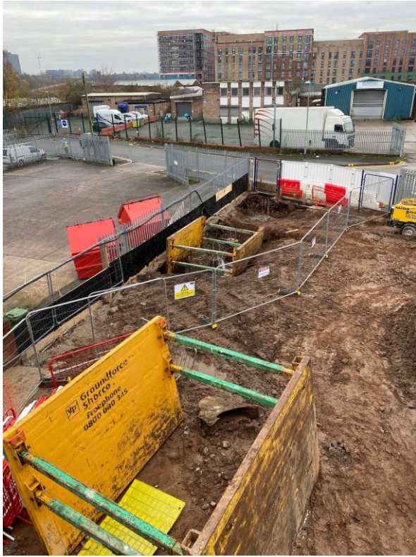
Block B – Temporary retaining structure onsite
