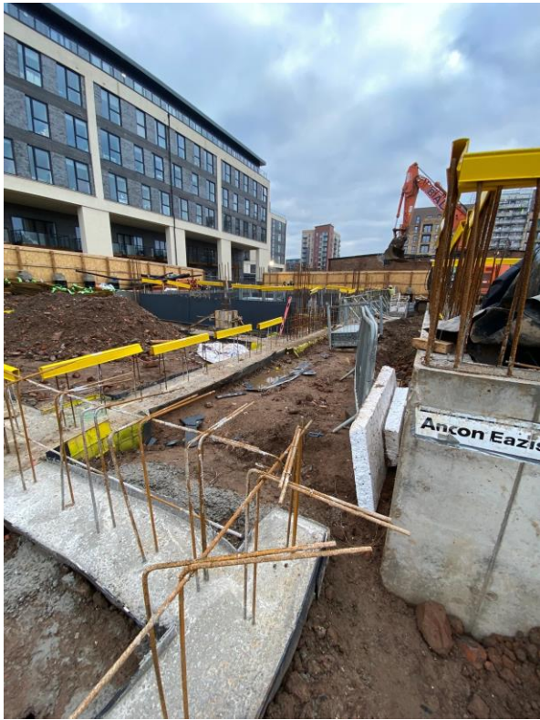
Block B – Capping beam in place
