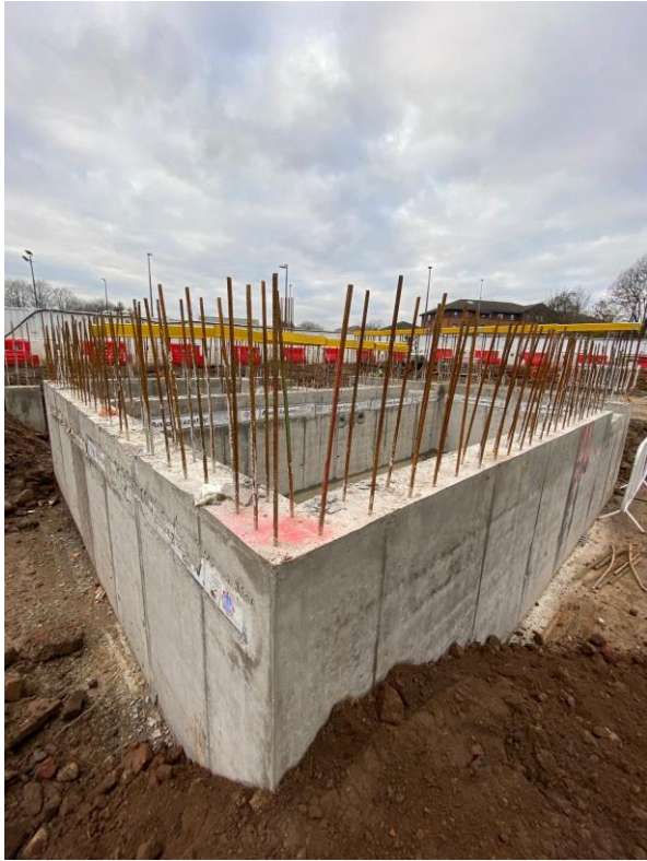
Lift core cast
