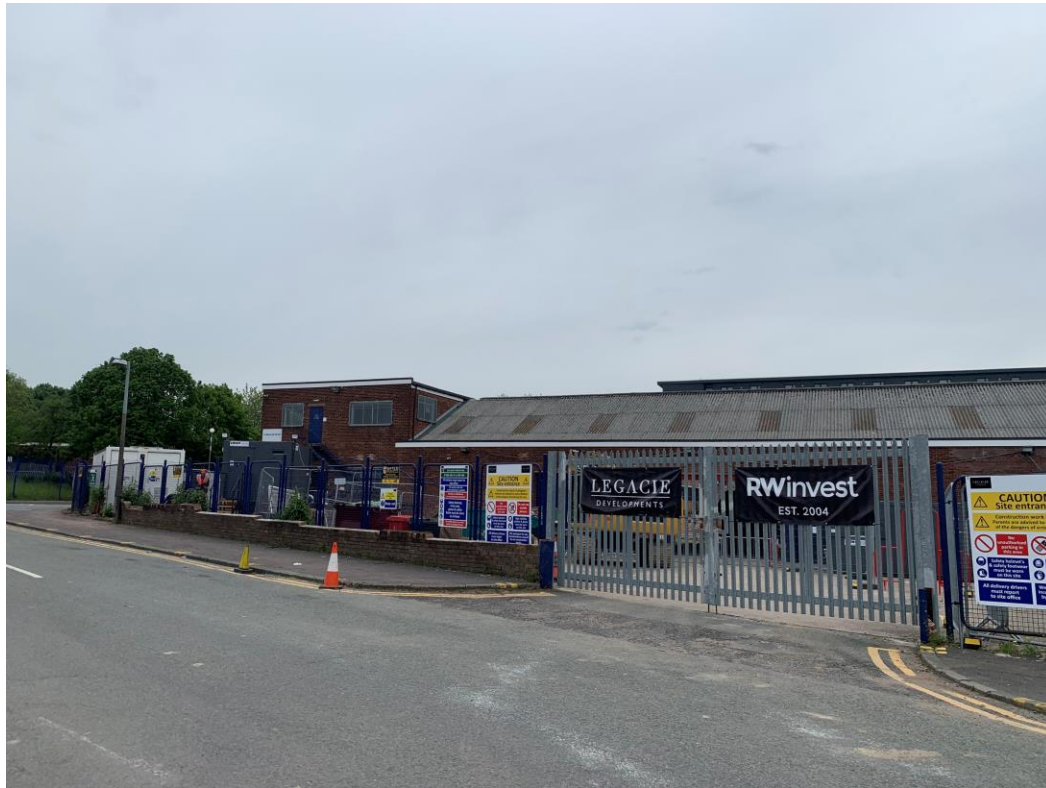
Worrall Street site view – buildings to be demolished
