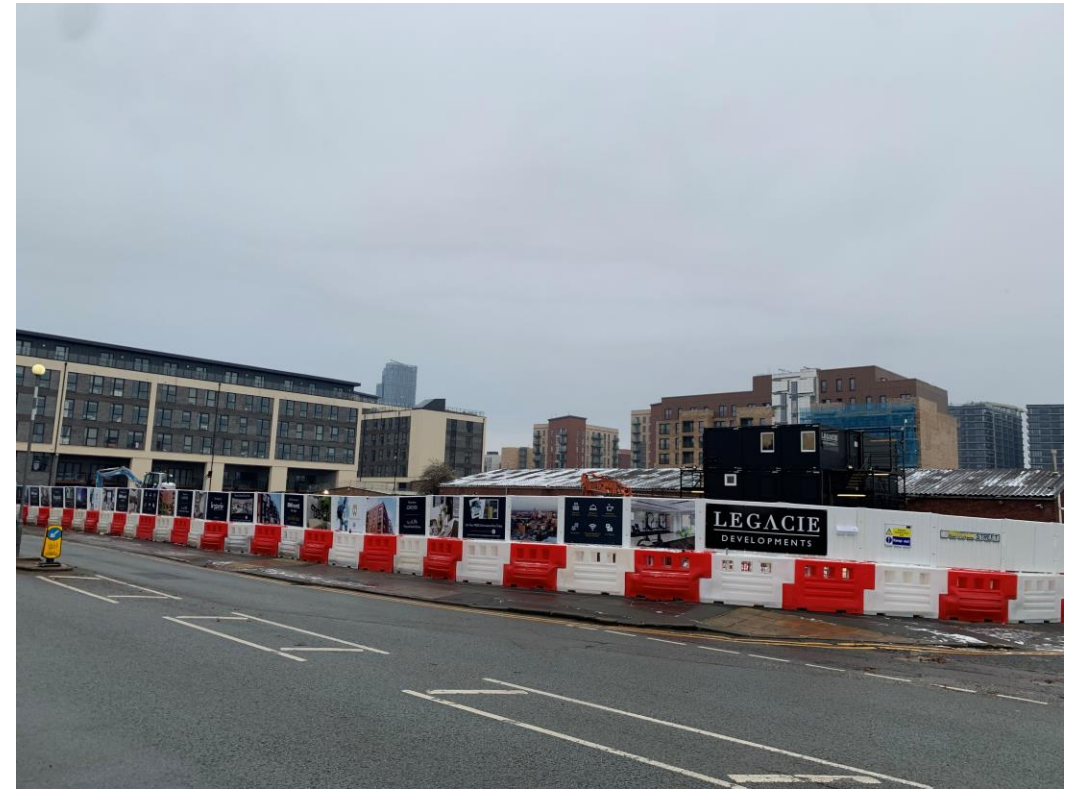
Ordsall Lane site view – buildings removed
