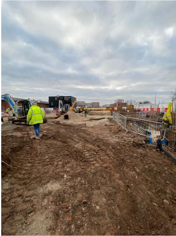
Site activity plant & machinery
