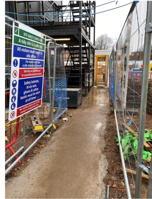
Block B – Turnstile site entrance
