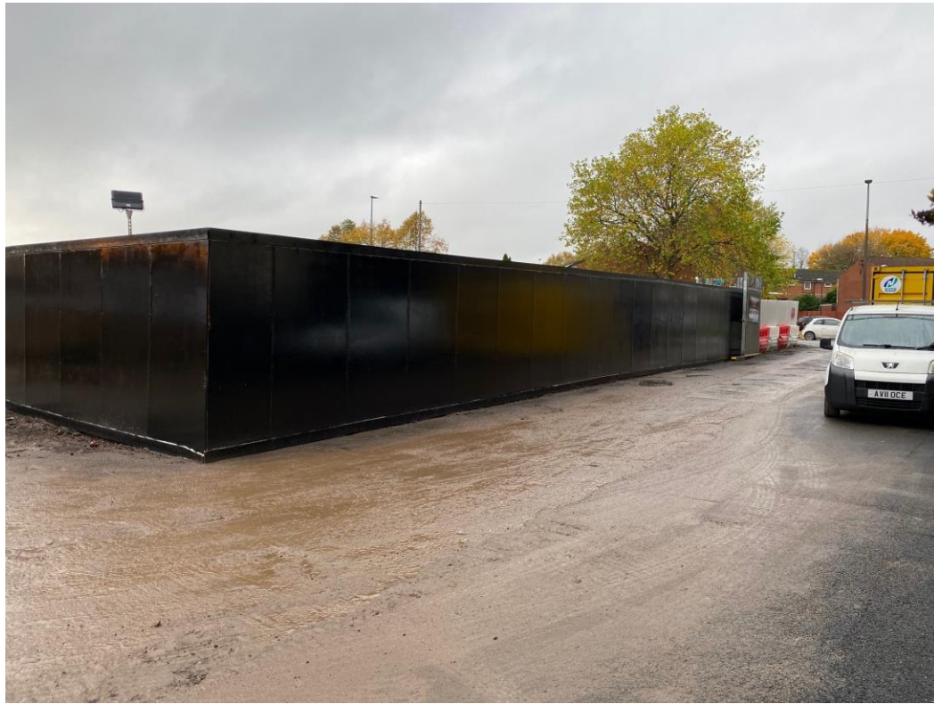
Worrall Lane site plant & deliveries entrance
