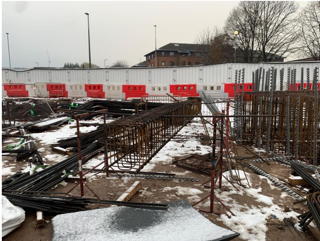
Foundation reinforcement cages being formed and stored
