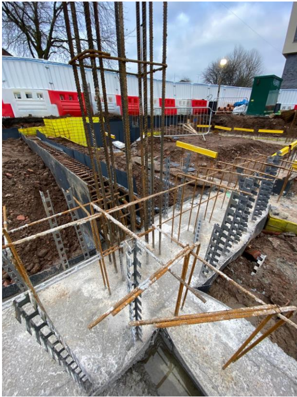
Block B – Capping beam in place
