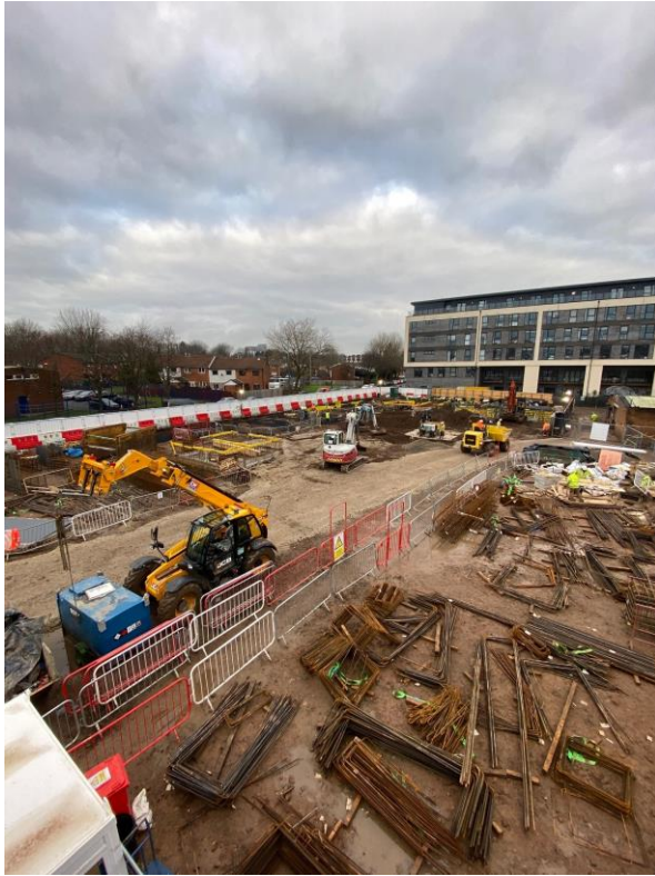
Site activity plant & machinery
