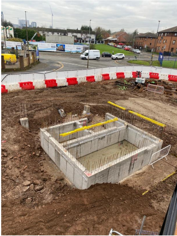
Core substructure installed
