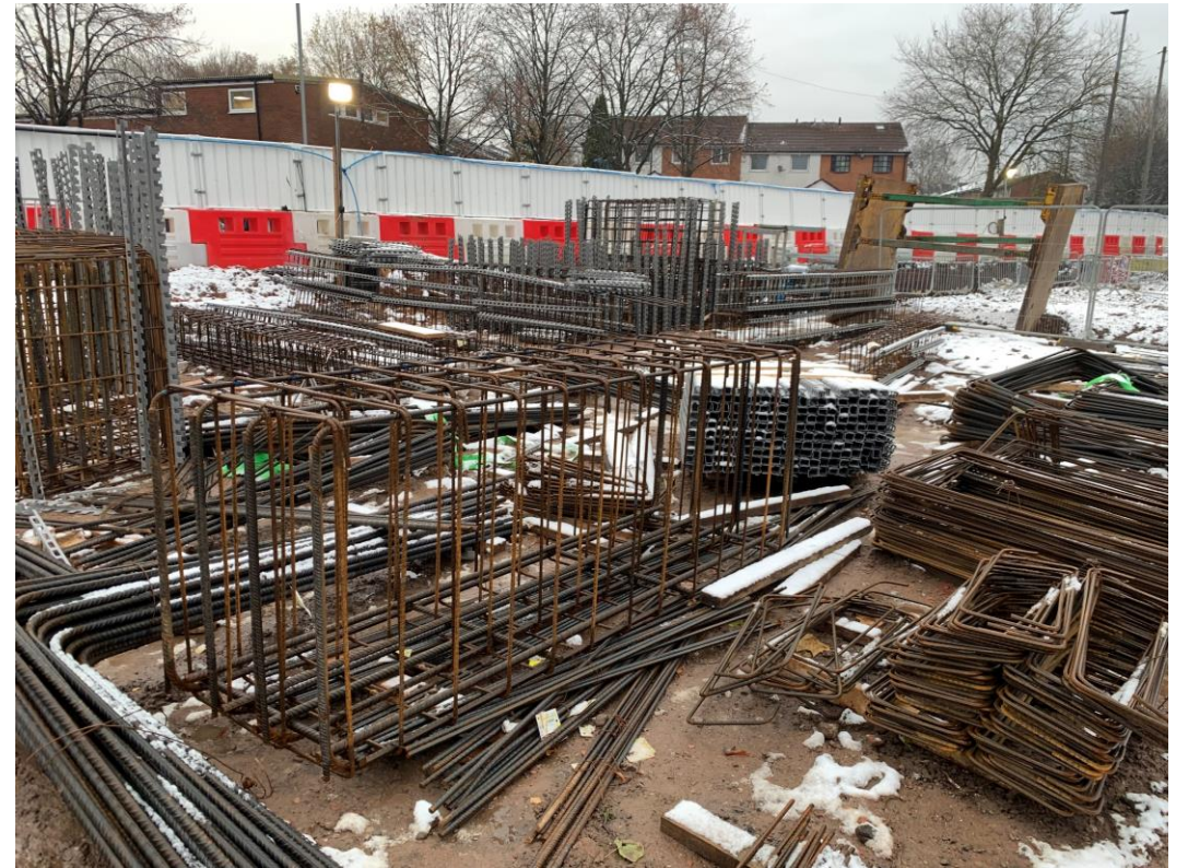
Foundation reinforcement cages being formed and stored
