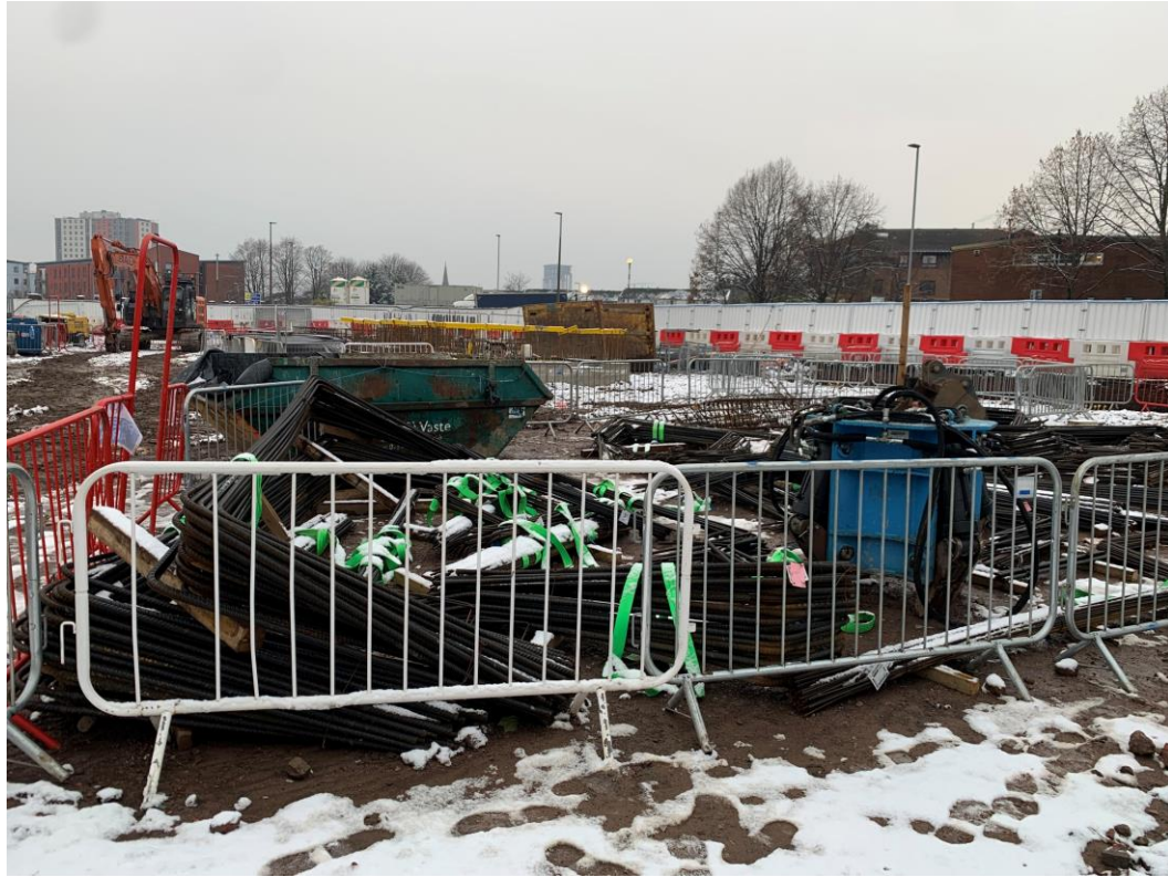
Foundation reinforcement stored
