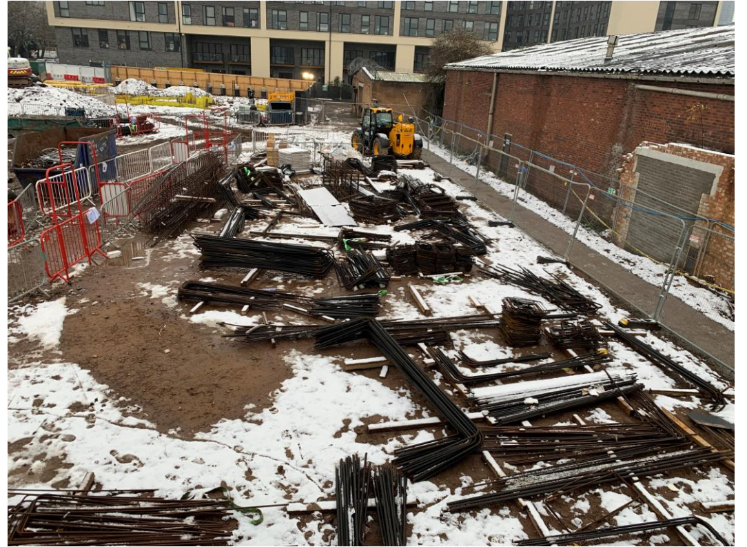
Foundation reinforcement stored
