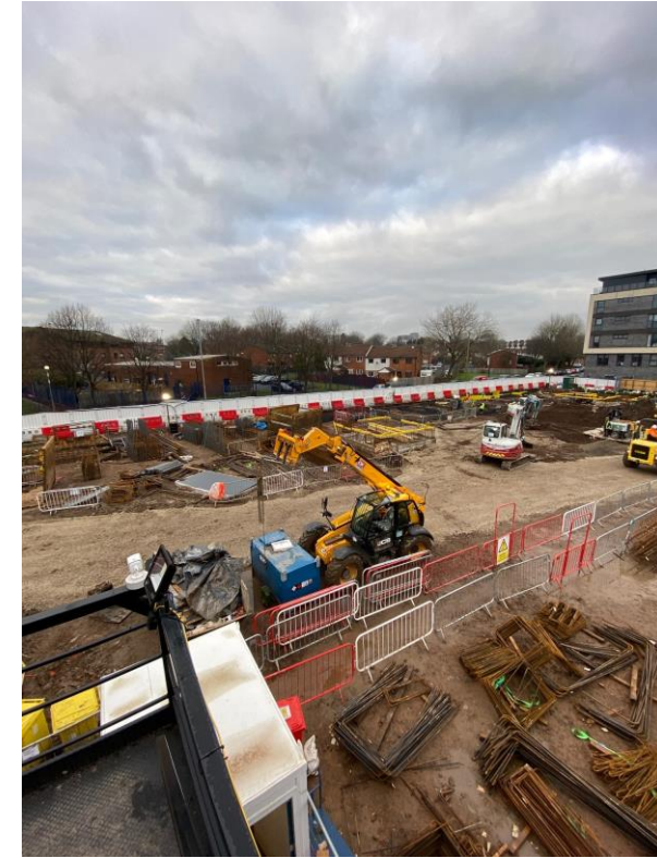
Site activity plant & machinery
