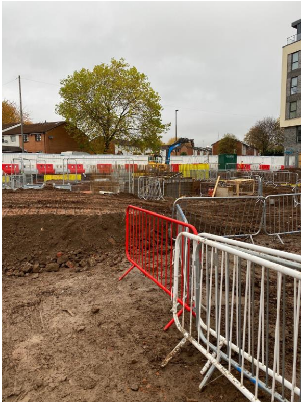
Site access barriers
