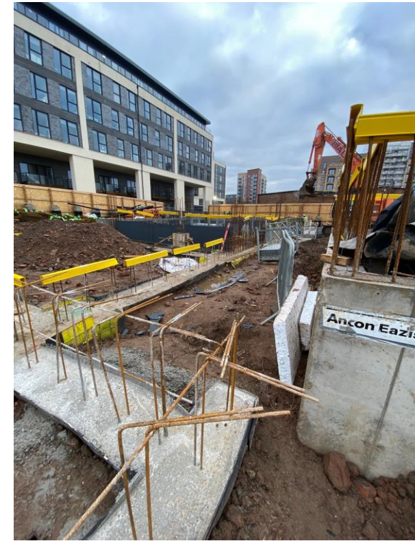
Block B – Capping beam in place
