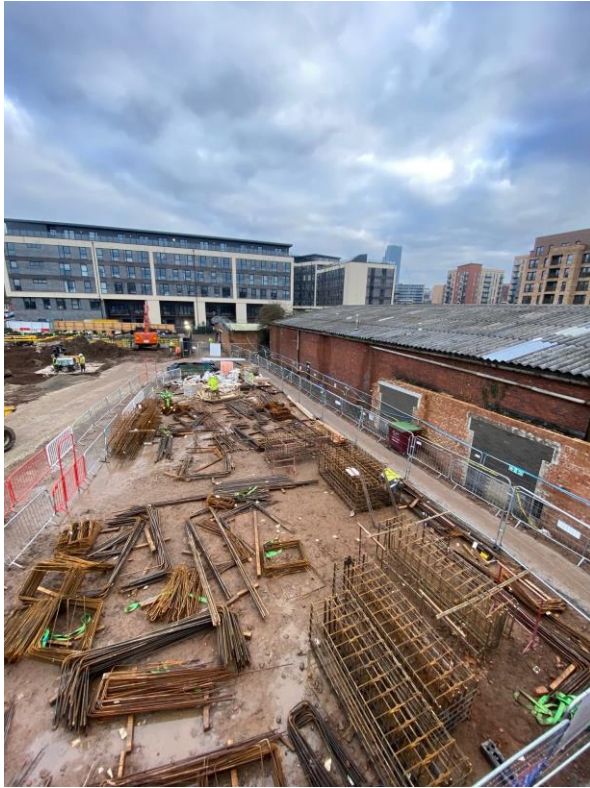
Foundation steel reinforcement stored
