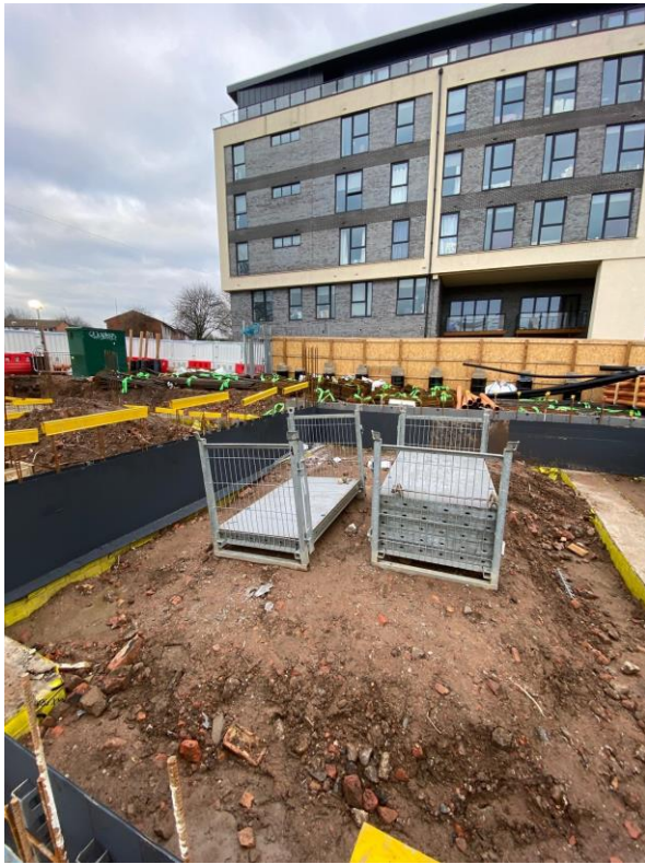
Steel shuttering onsite
