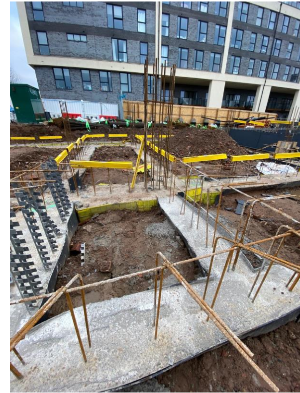
Block B – Capping beam in place
