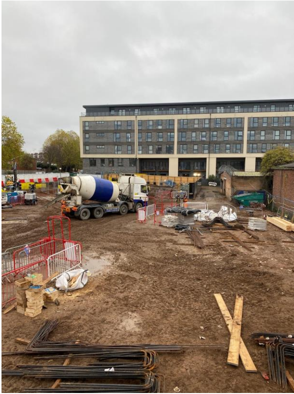
Foundation reinforcement stored
