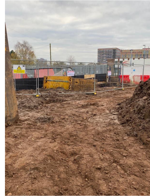
Hoardings & barriers in place
