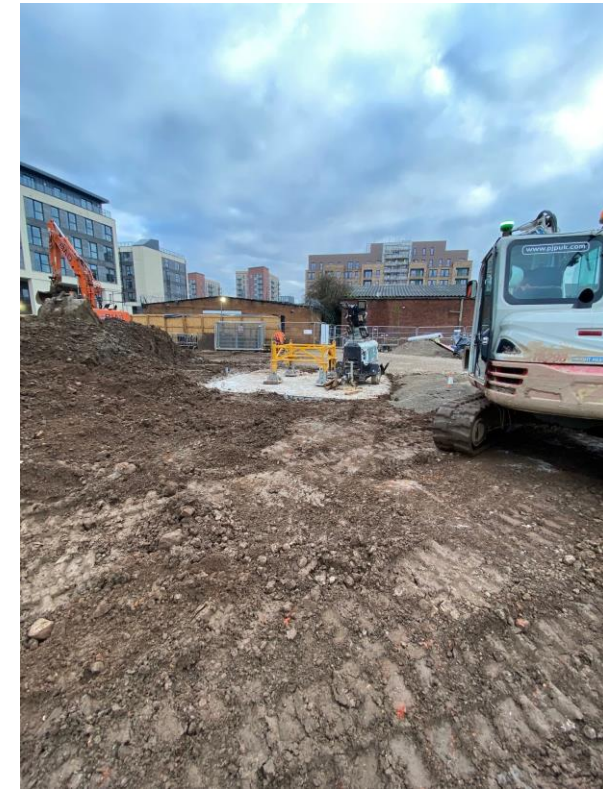
Crane base installed
