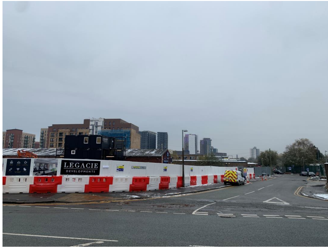
Ordsall Lane site view – buildings removed
