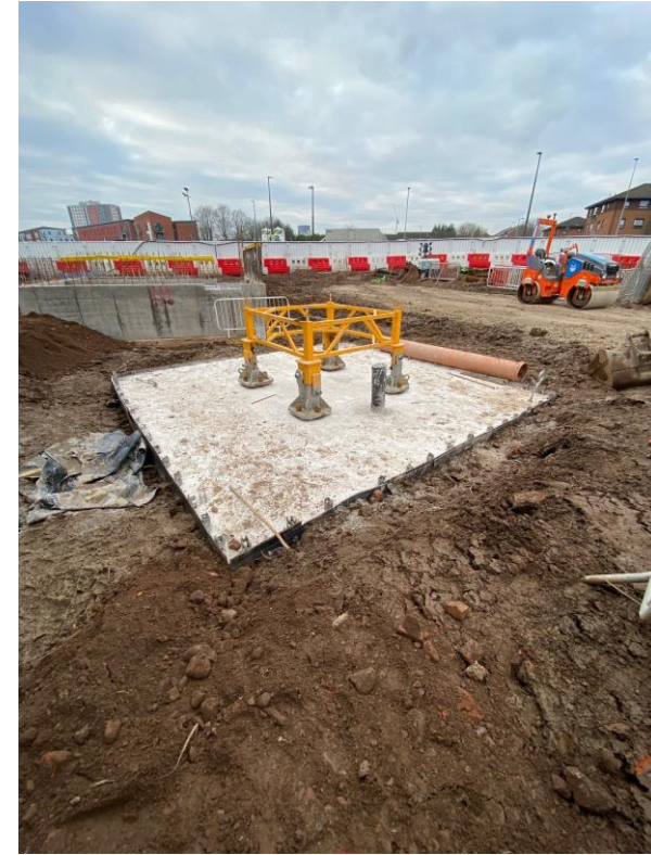
Core substructure installed
