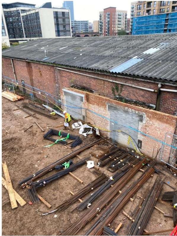
Foundation reinforcement stored
