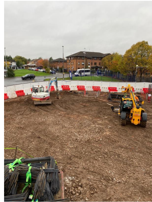
Site activity plant and machinery
