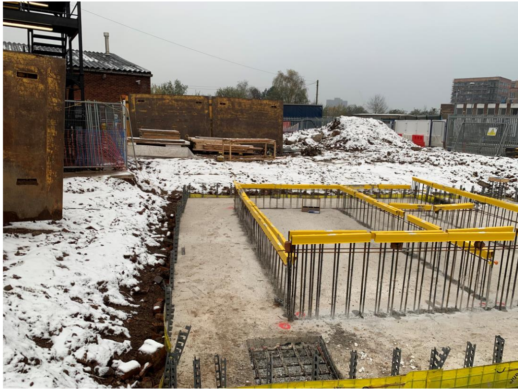
Block A - Core substructure
