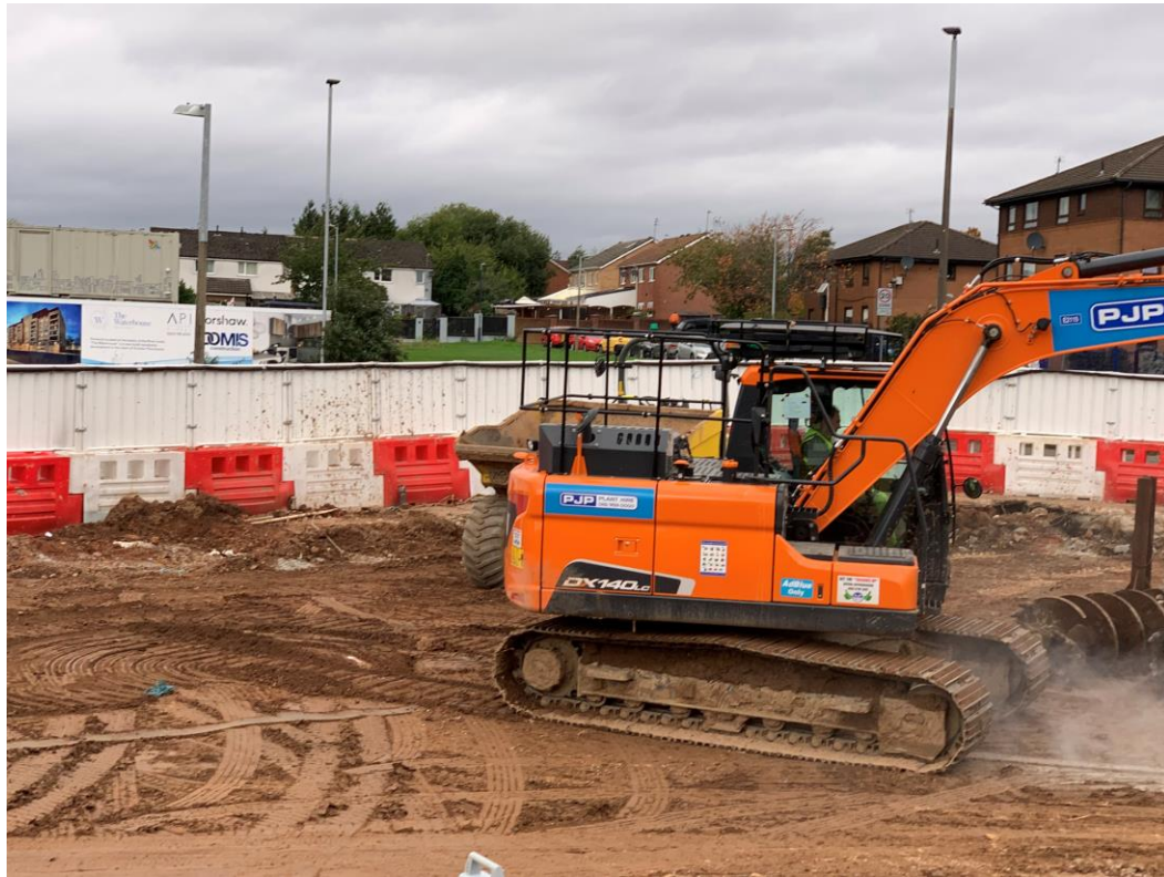
Site activity plant and machinery
