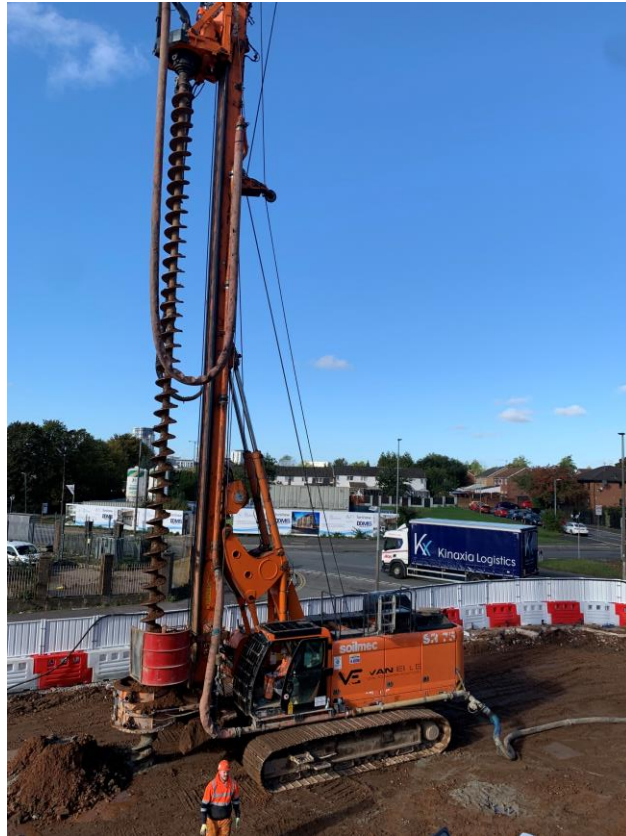
Rotary bored piling rig
