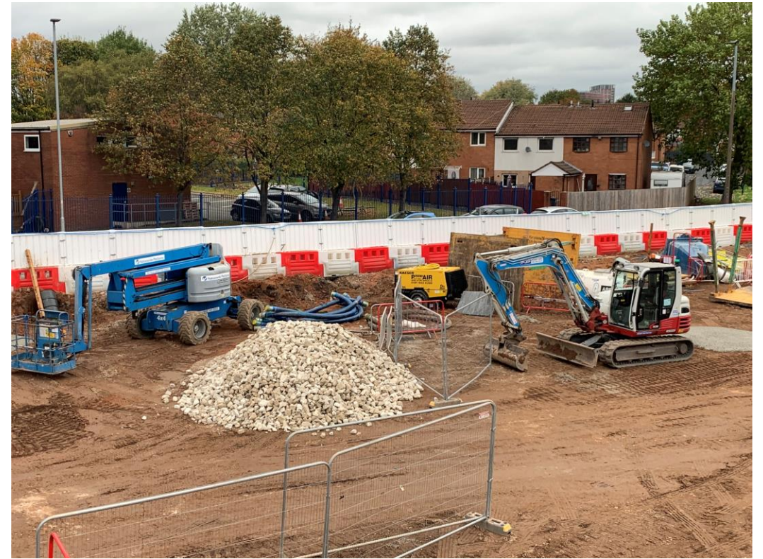
Steel reinforcement foundation cages being fabricated
