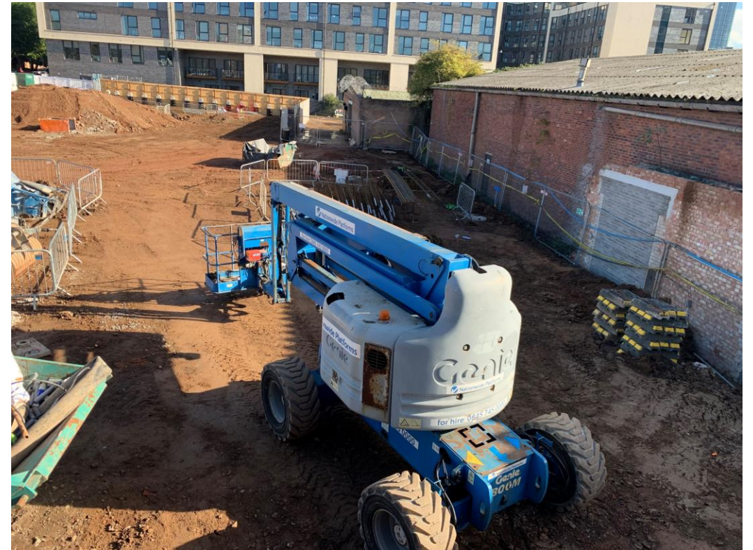
Site activity plant and machinery
