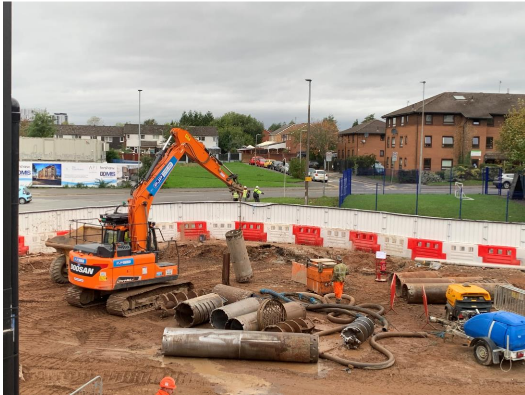
CFA piling rig components cleaning process
