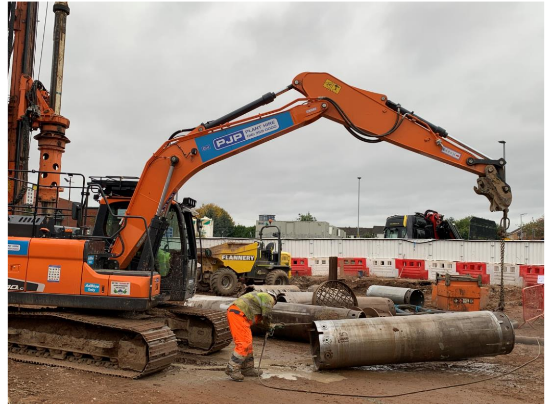
CFA piling rig components cleaning process
