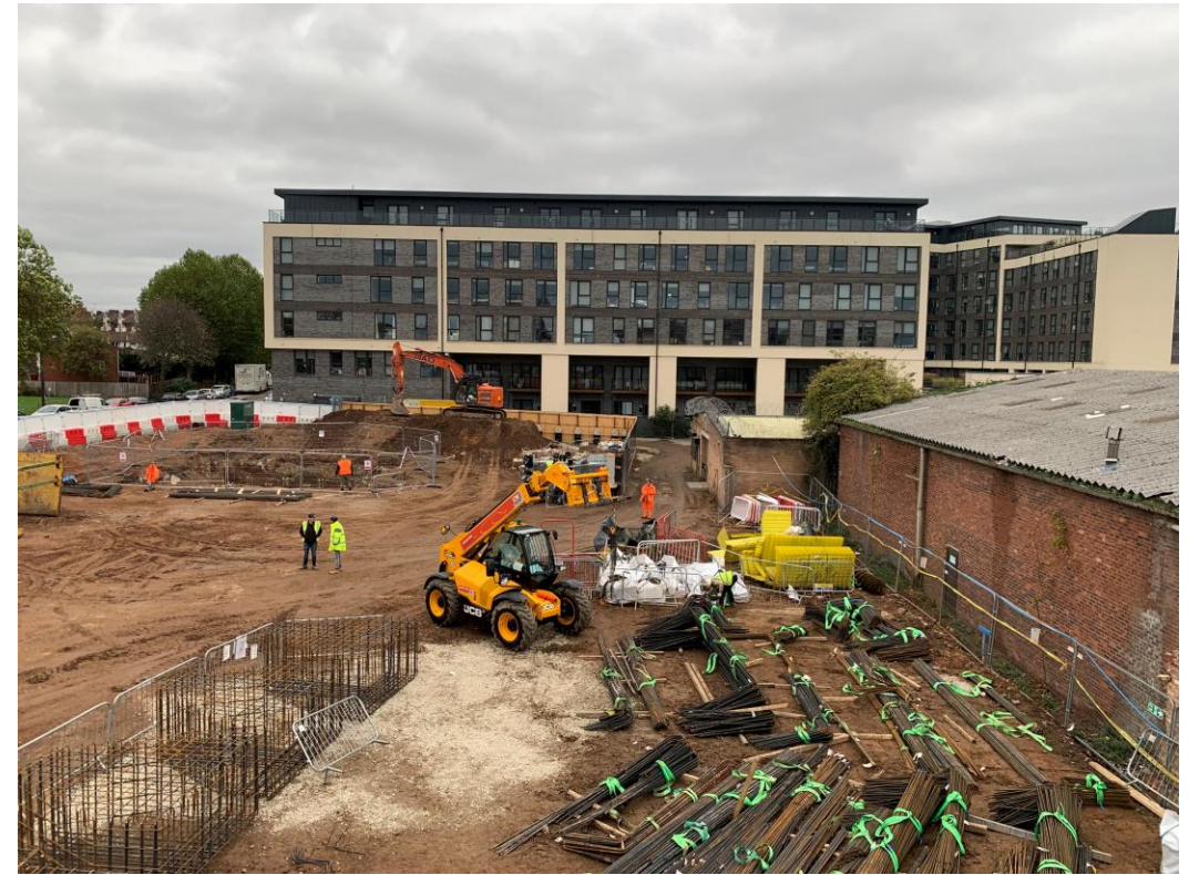
Steel reinforcement foundation cages being fabricated
