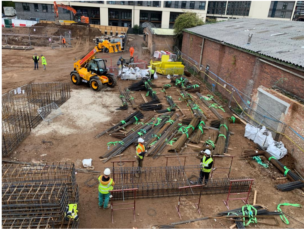
Steel reinforcement foundation cages being fabricated
