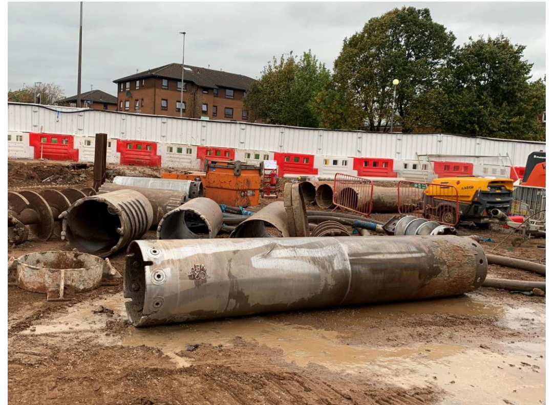
CFA piling rig components cleaning process
