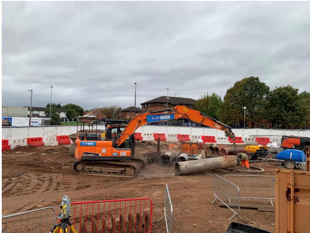
CFA piling rig components cleaning process
