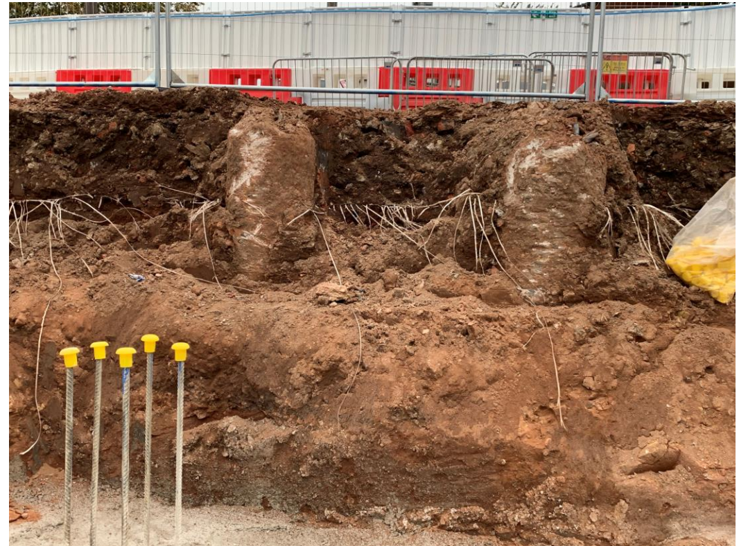
Completed piles exposed
