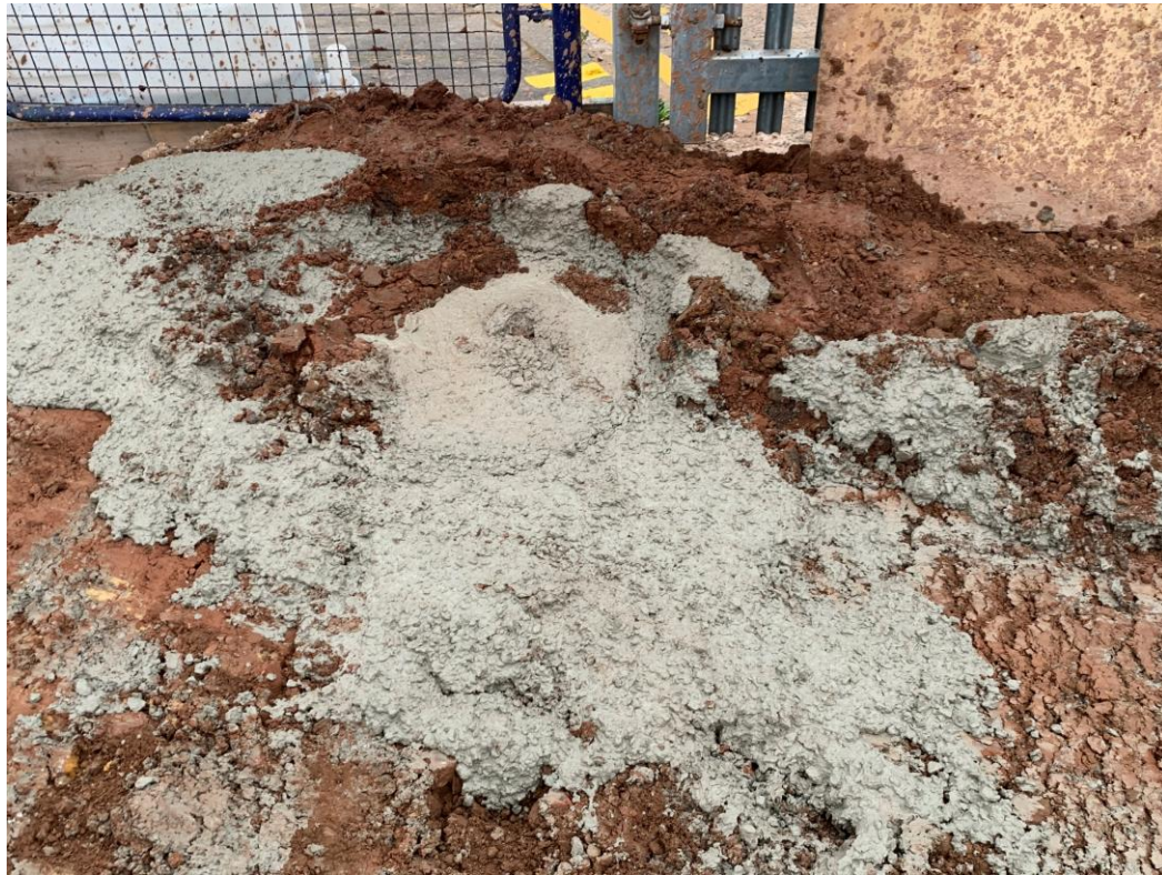
Last CFA pile complete today
