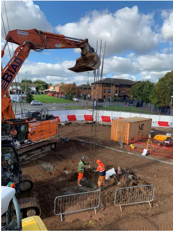
Piling cage reinforcement installed
