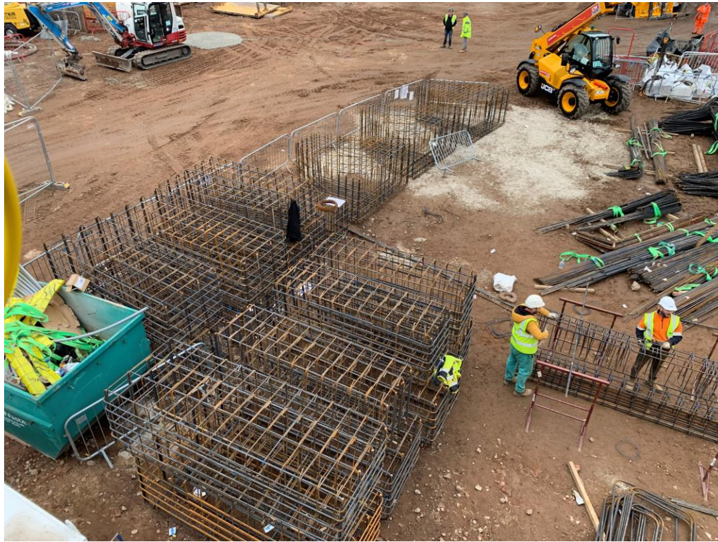
Steel reinforcement foundation cages being fabricated
