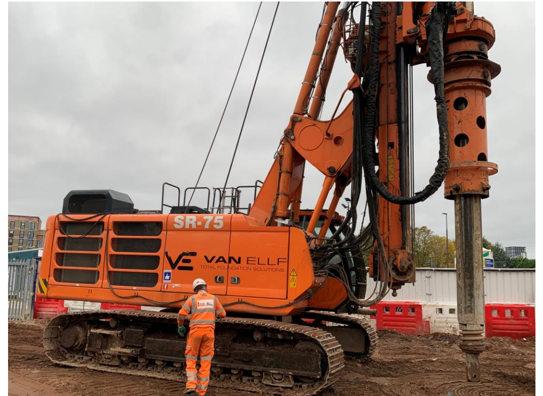
CFA piling rig
