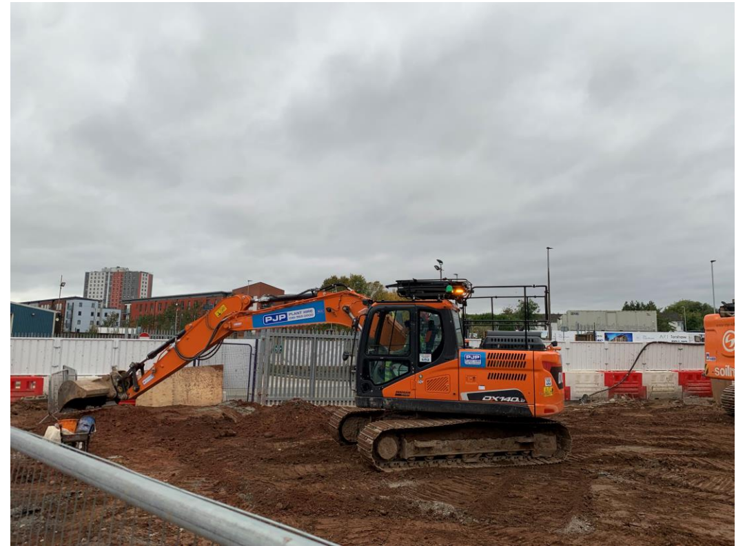
Site activity plant and machinery
