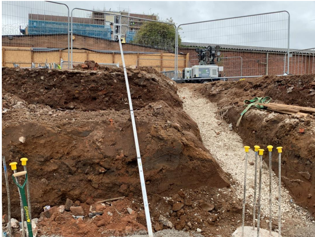
Tower crane pad access
