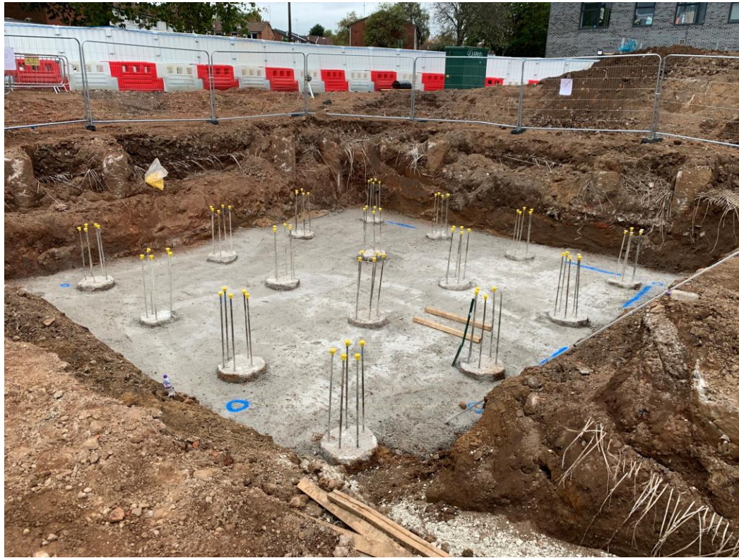
Tower crane pad under construction
