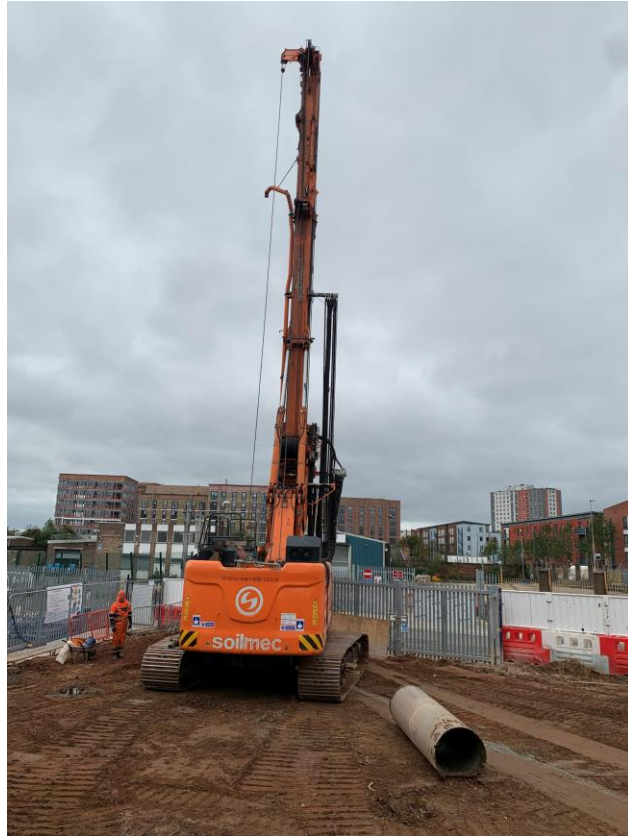
CFA piling rig
