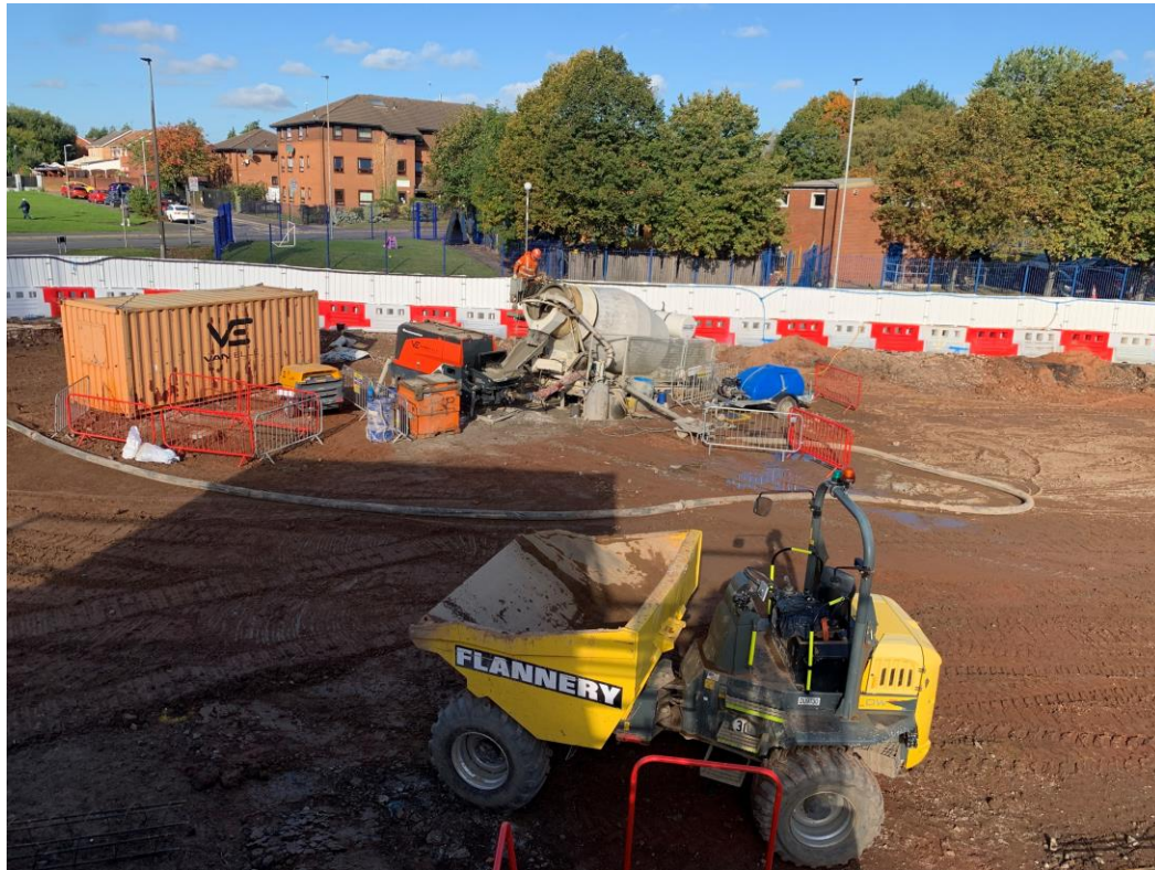
Site activity plant and machinery
