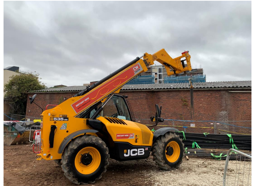
Site plant and machinery
