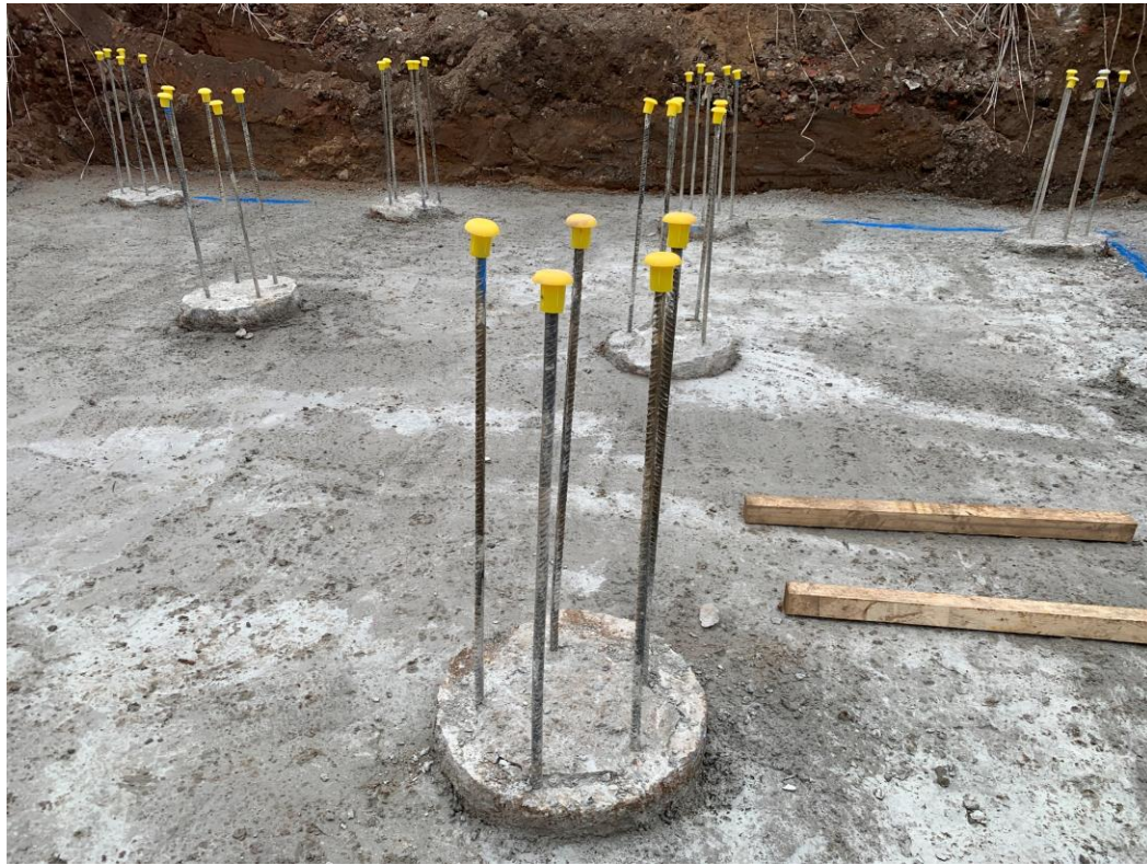
Piling capping commenced
