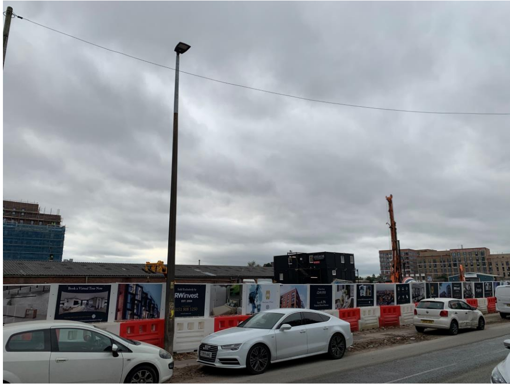
Ordsall Lane site view – buildings removed
