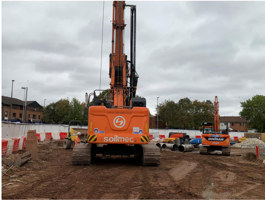
CFA piling rig
