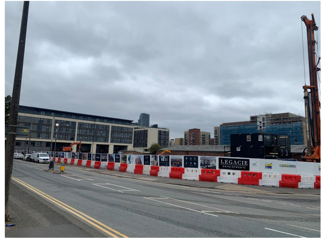
Ordsall Lane site view – buildings removed
