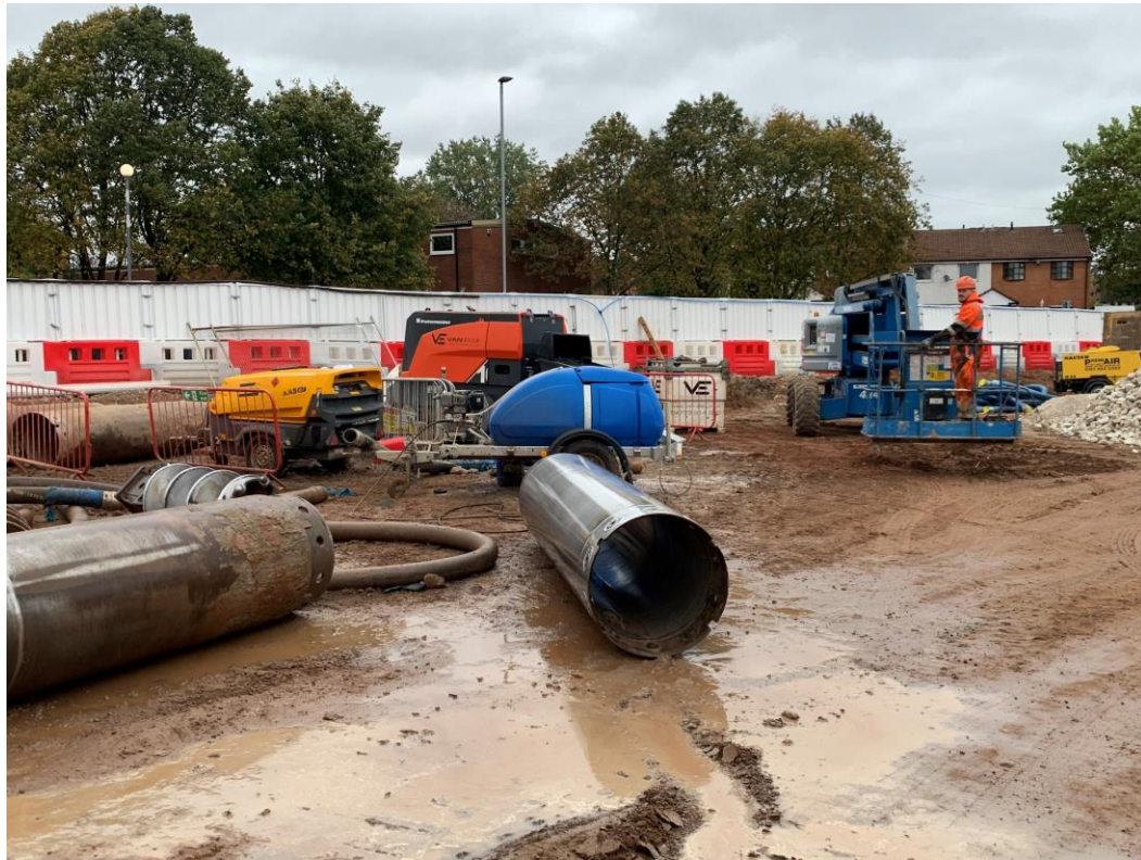
CFA piling rig components cleaning process
