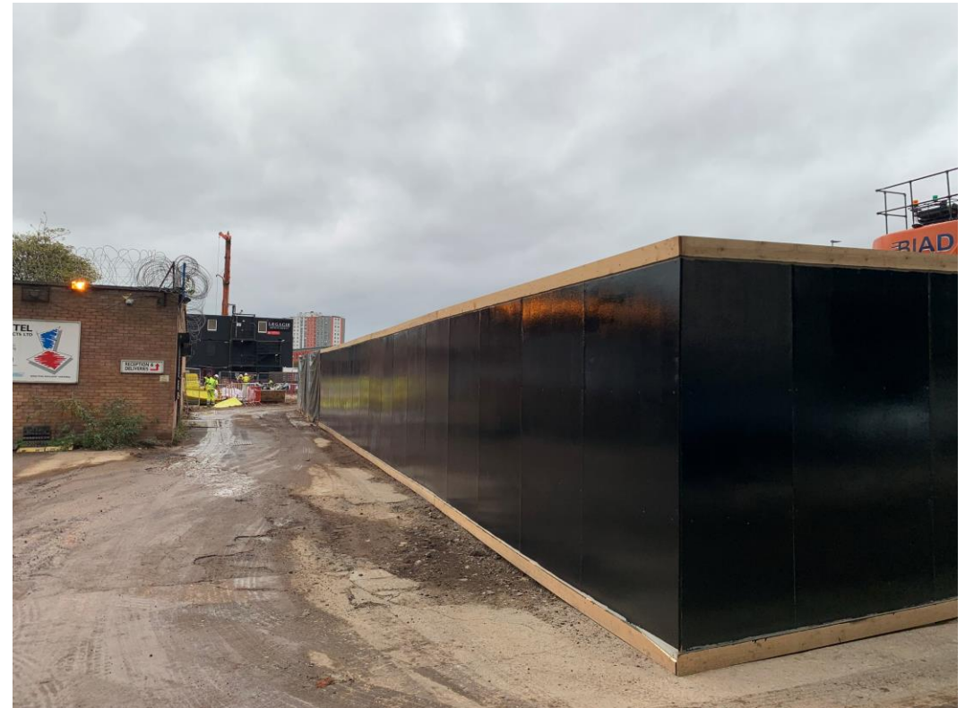
Worral Lane site plant & deliveries entrance
