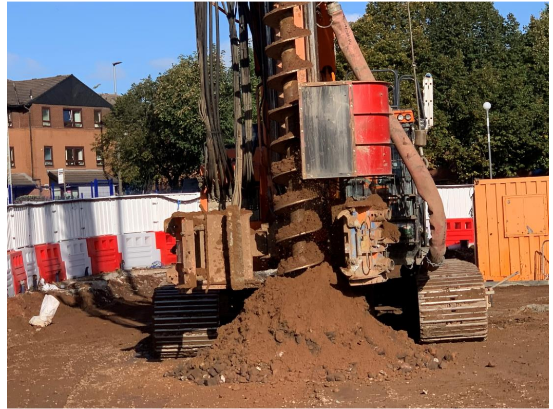
Rotary bored piling
