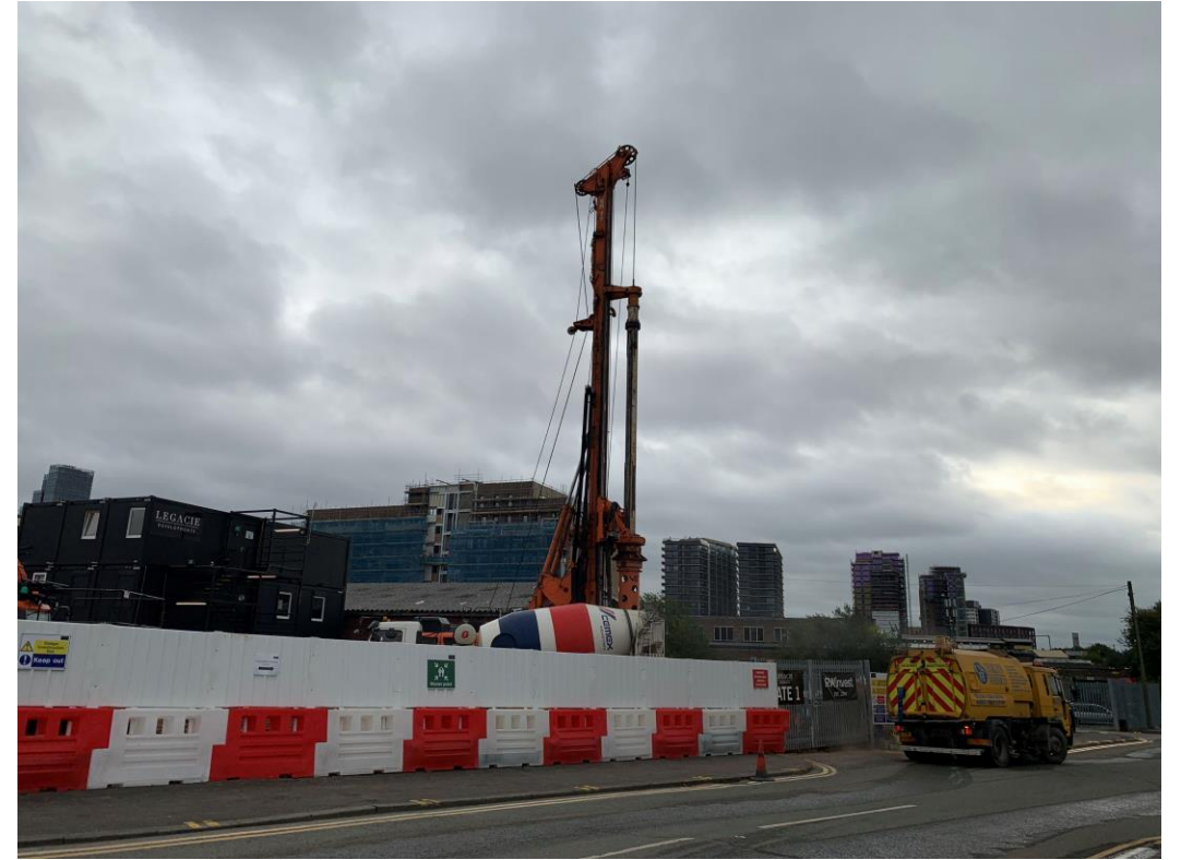
Ordsall Lane site view – buildings removed
