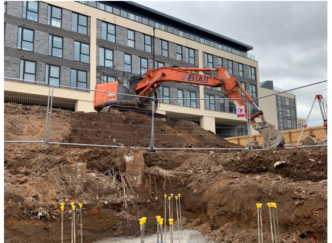
Site excavation works
