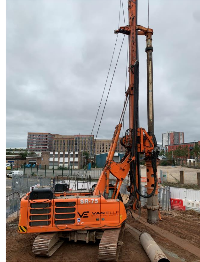
CFA piling rig
