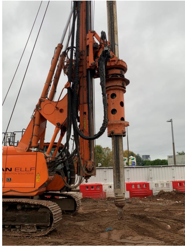
CFA piling rig
