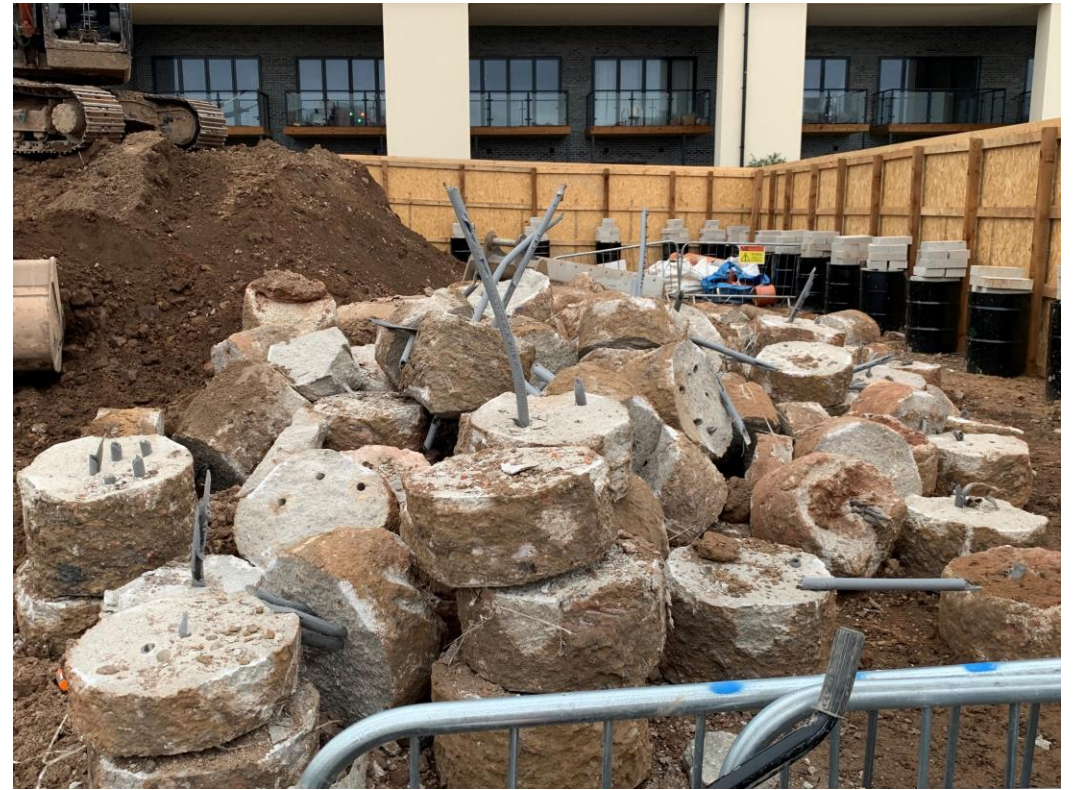
Piling tops removed
