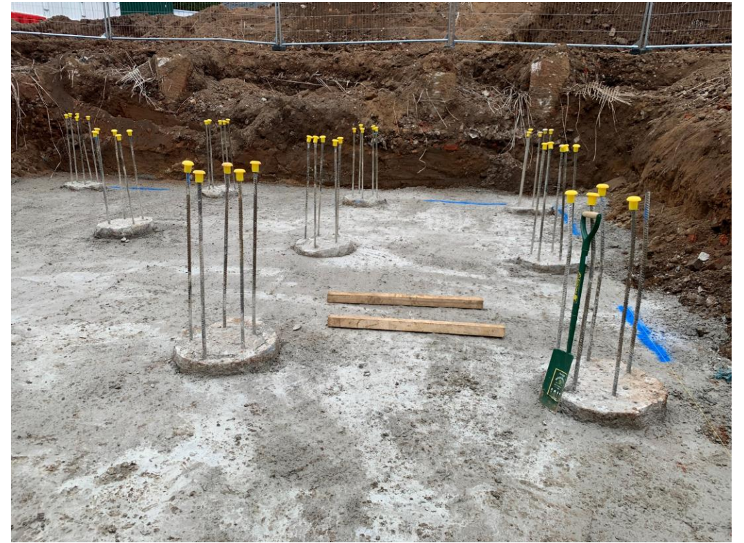
Tower crane pad under construction
