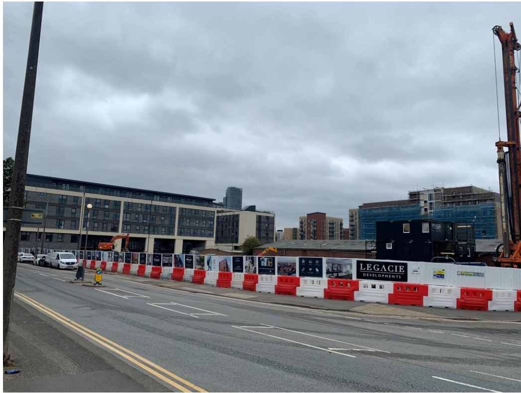
Ordsall Lane site view – buildings removed
