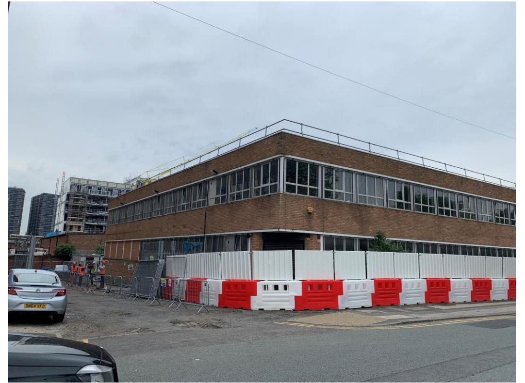
Ordsall Lane site view – buildings to be demolished
