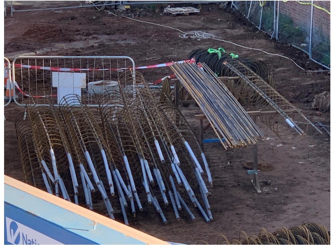
Piling cage reinforcement
