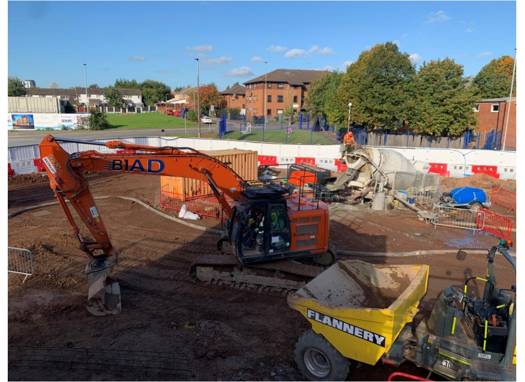
Site activity plant and machinery
