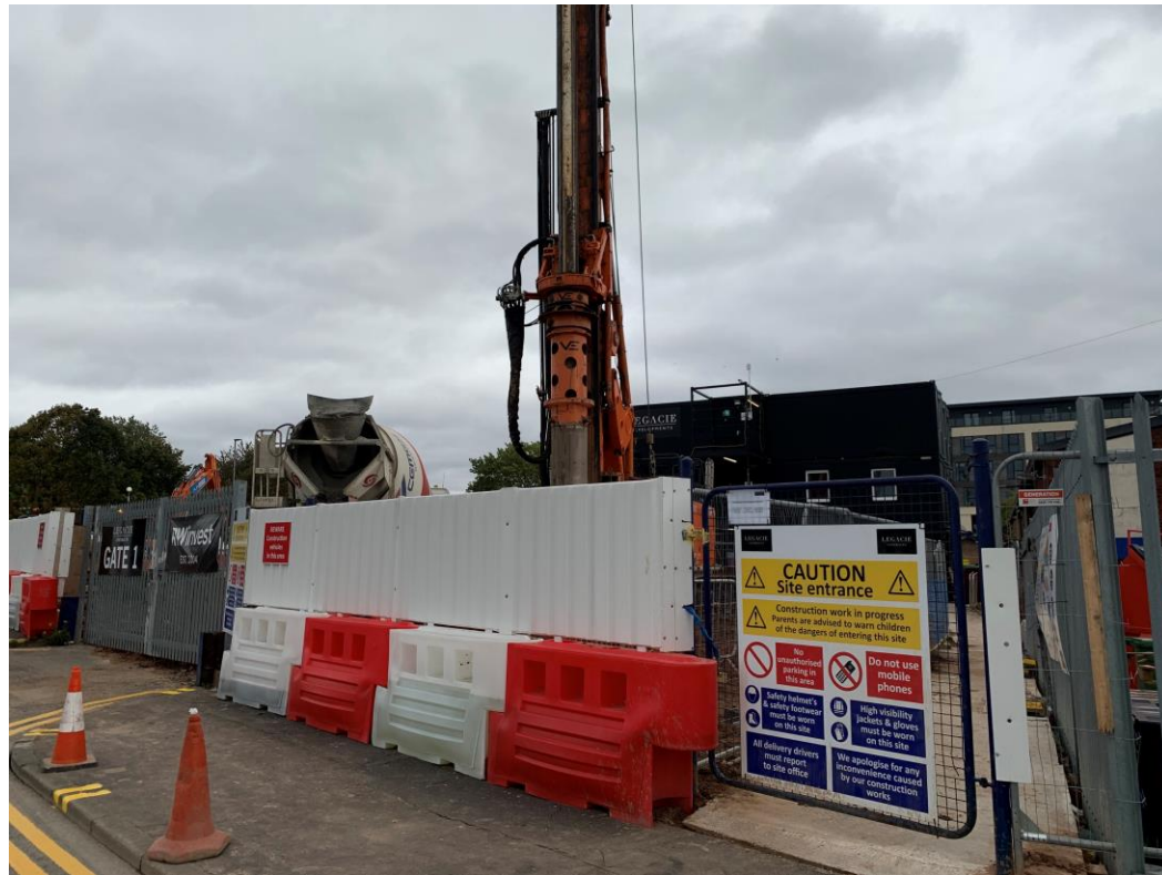
Worral Lane site pedestrian entrance
