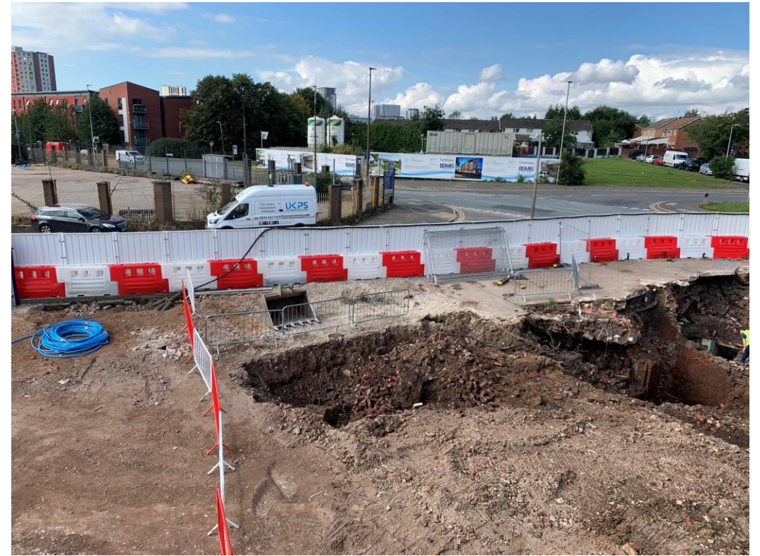
Site activity site formation levelling
