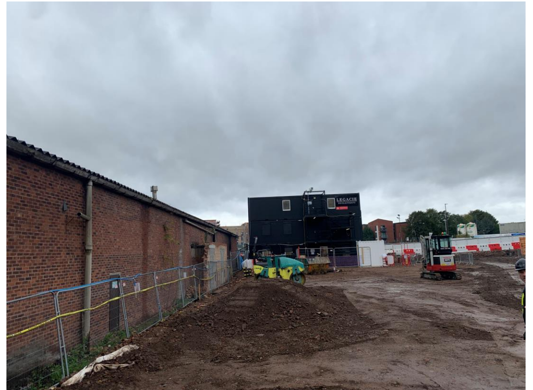
Site activity site formation piling mat
