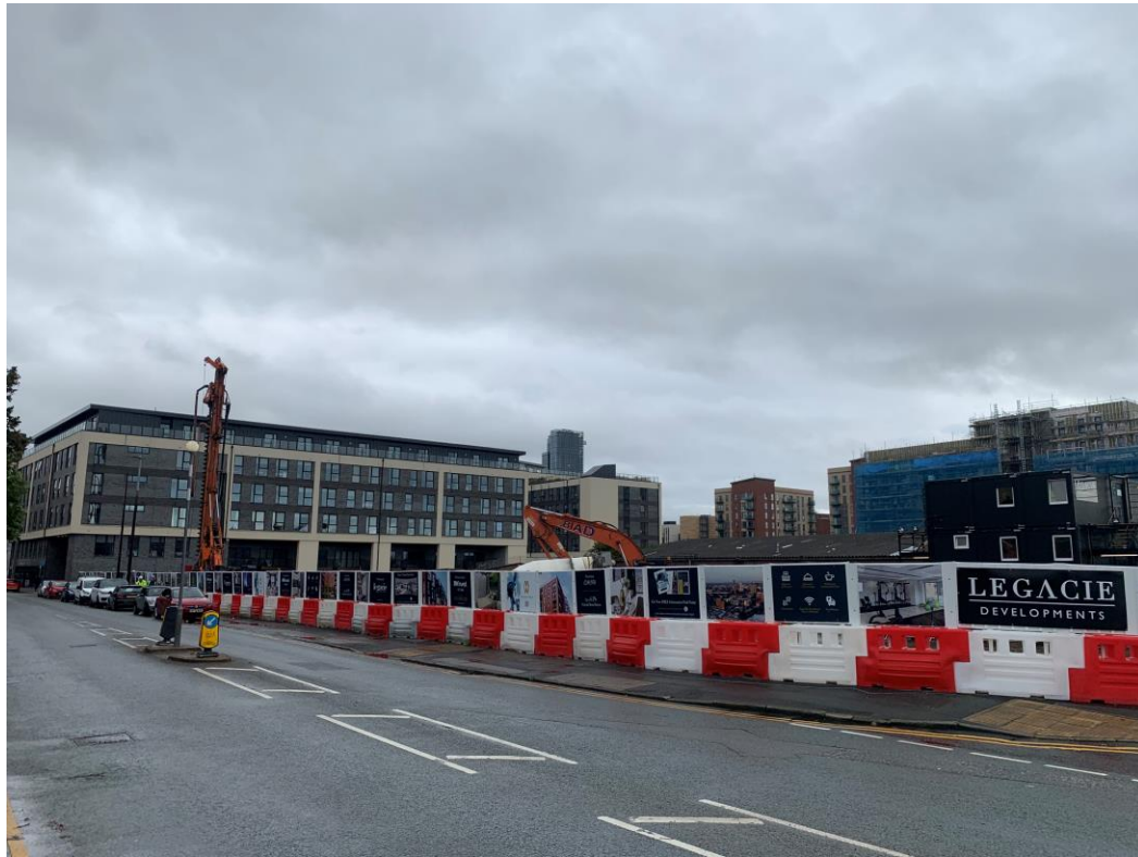
Ordsall Lane site view – buildings removed
