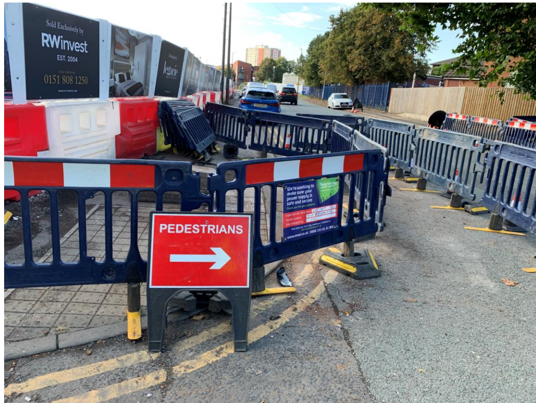
Ordsall Lane site view – buildings removed
