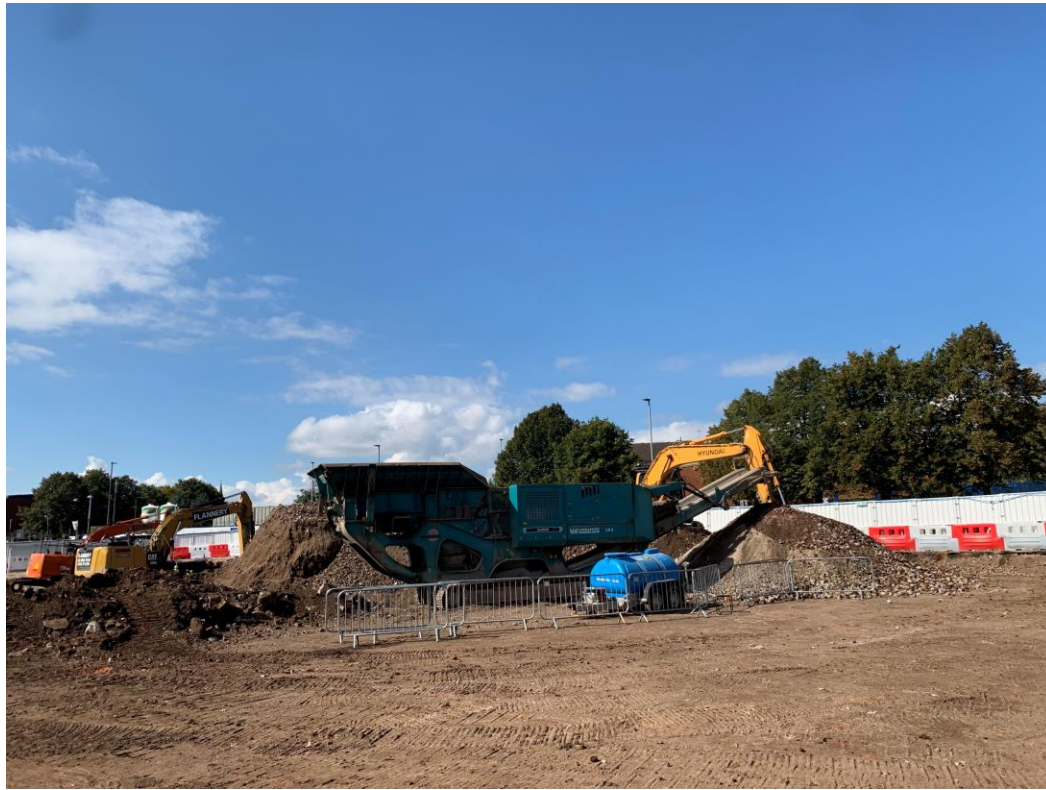
Site activity site levelling and stock piling
