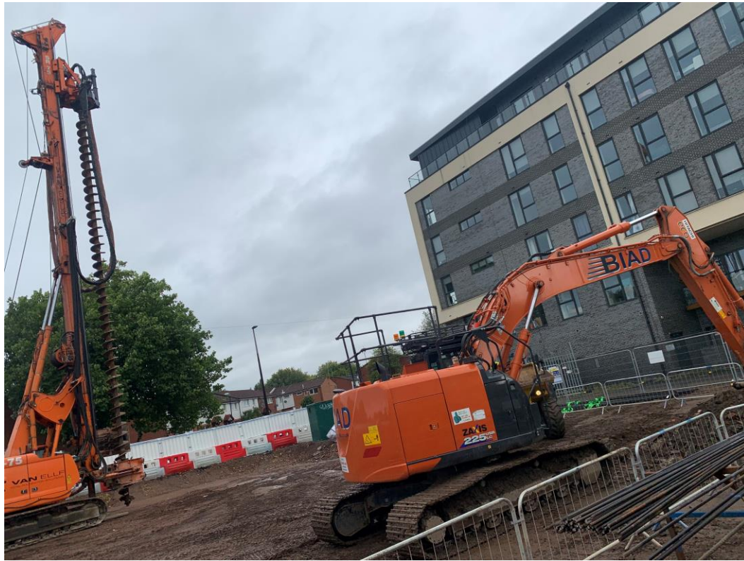
Site activity site plant and machinery
