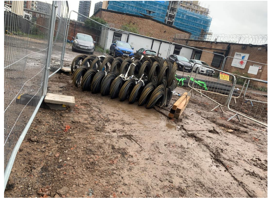
Piling cage reinforcement
