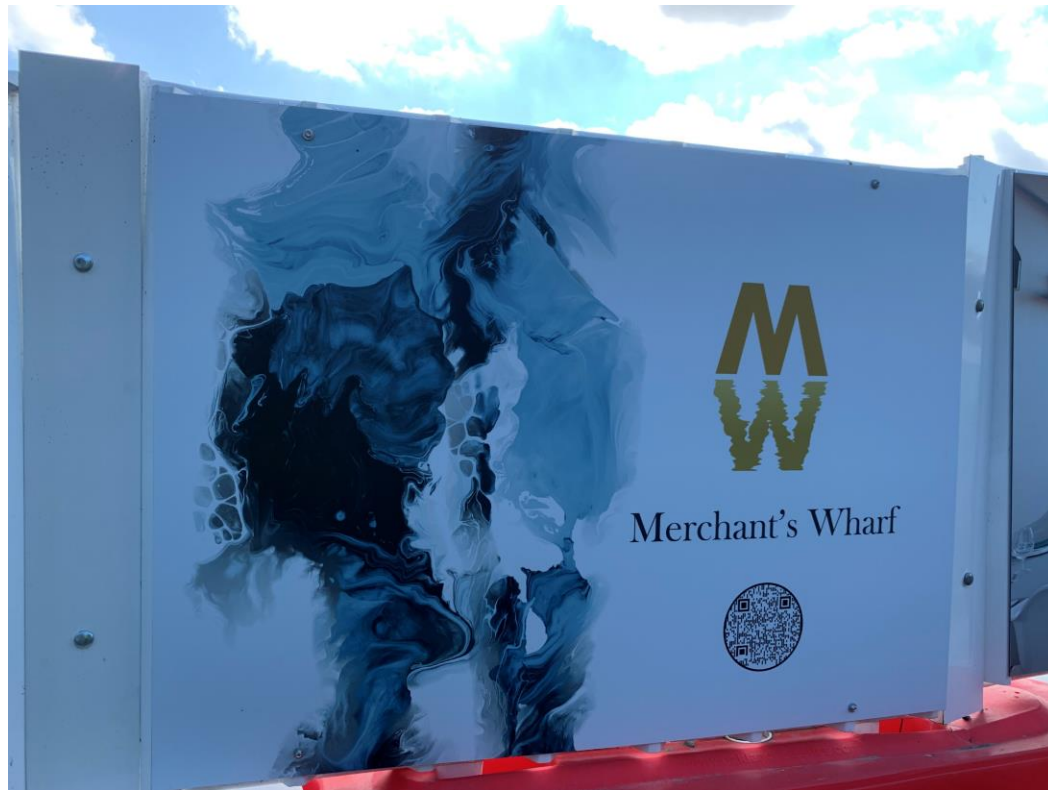
Ordsall Lane site view – site hoardings
