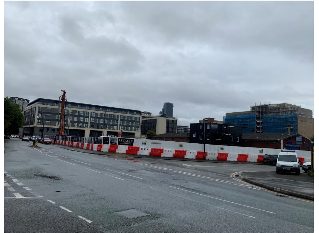
Ordsall Lane site view – buildings removed
