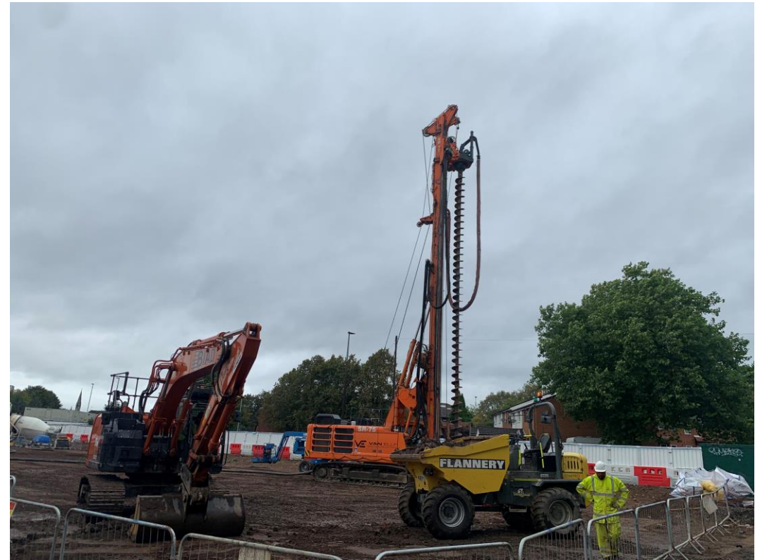
Site activity site plant and machinery
