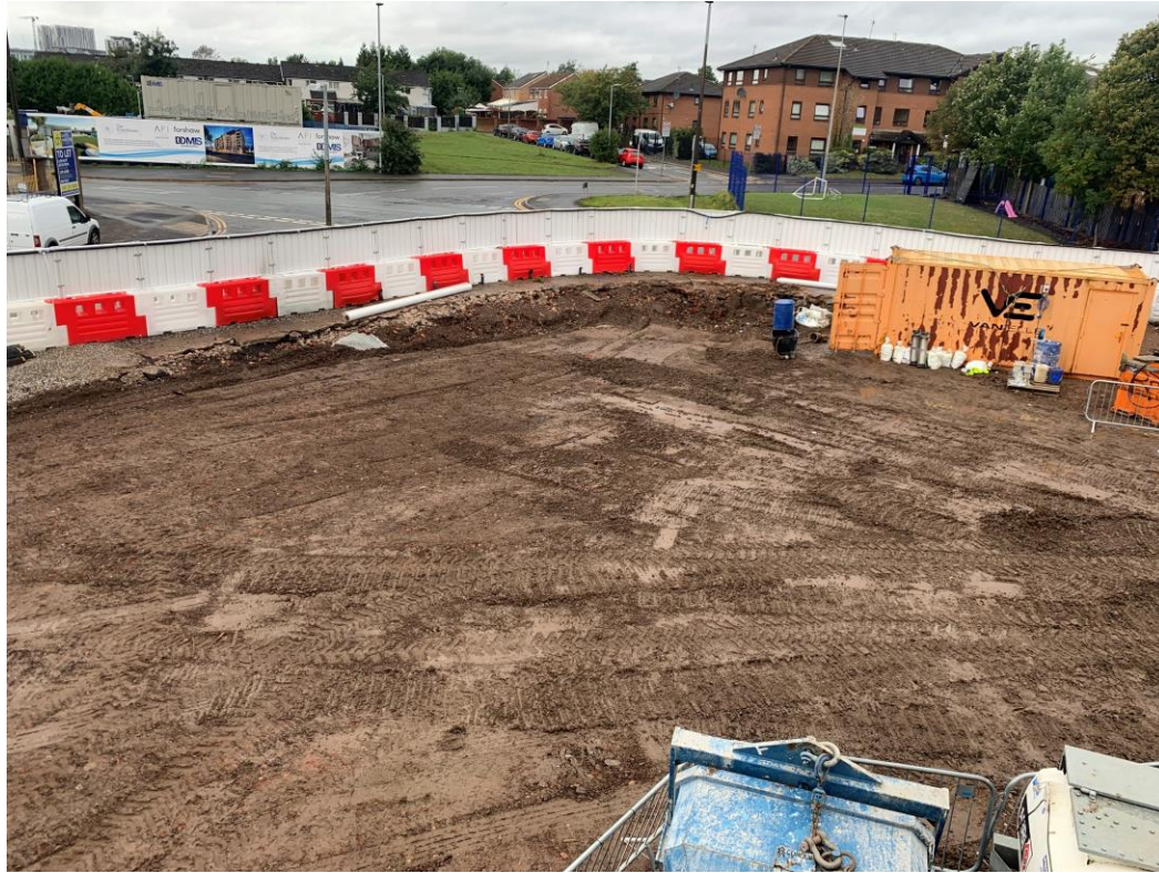
Site activity site formation piling mat
