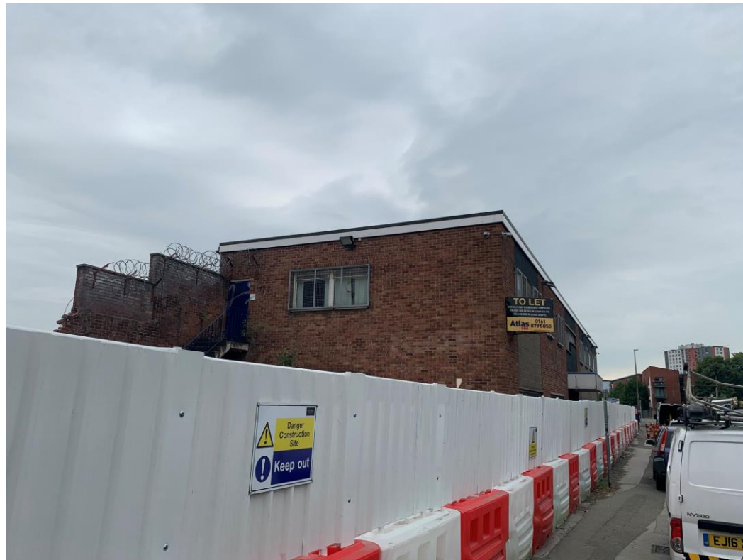
Ordsall Lane site view – buildings demolished
