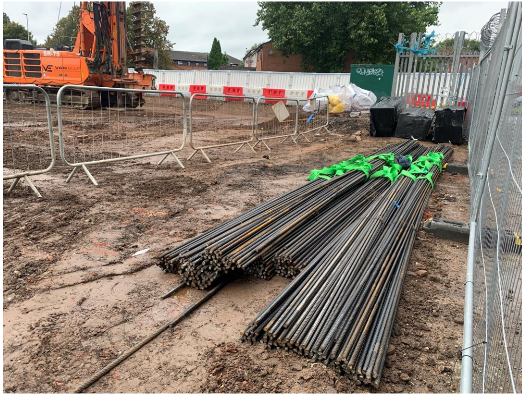
Piling cage reinforcement
