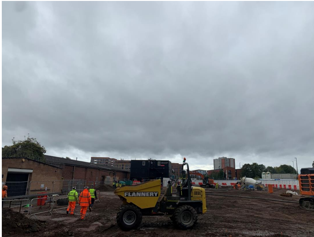
Site activity site formation piling mat
