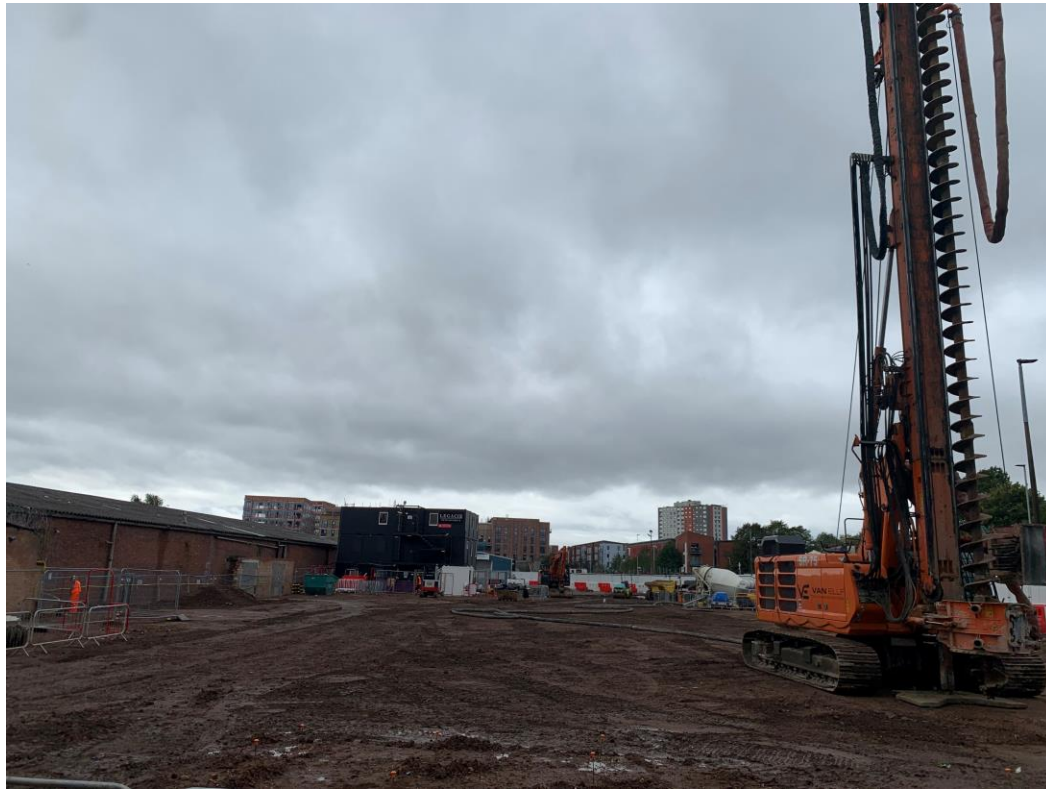
Site activity site formation piling mat
