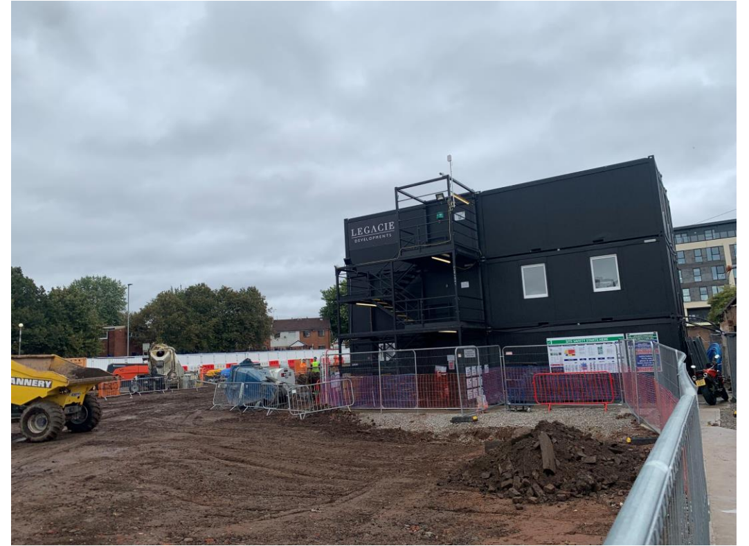
Site activity site formation piling mat
