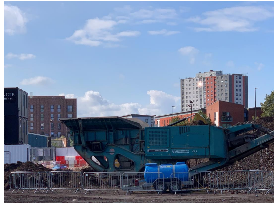
Site plant material crusher
