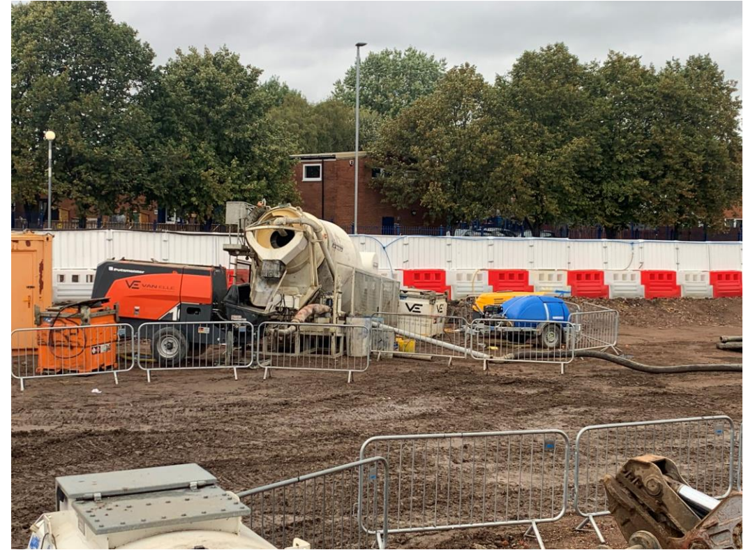
Site activity site formation piling mat
