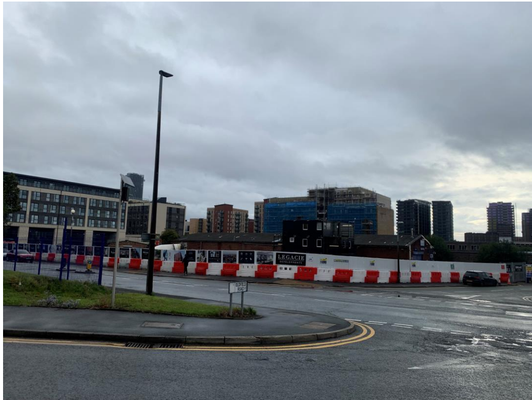
Ordsall Lane site view – buildings removed
