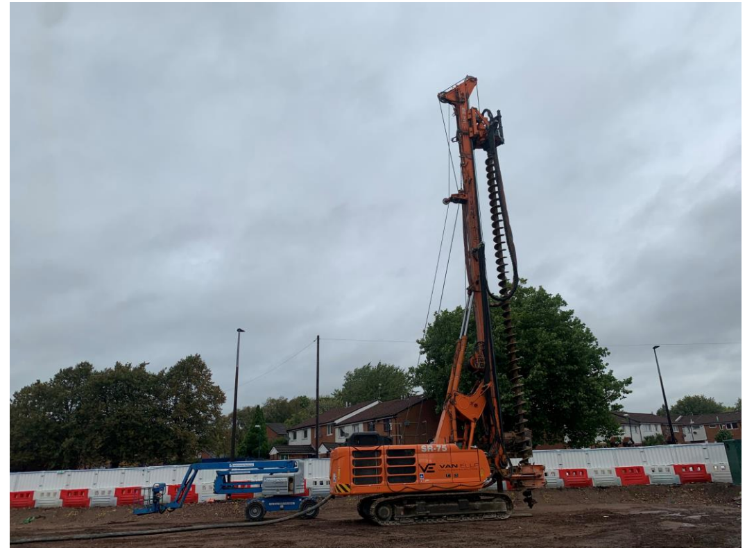
Auger piling rig
