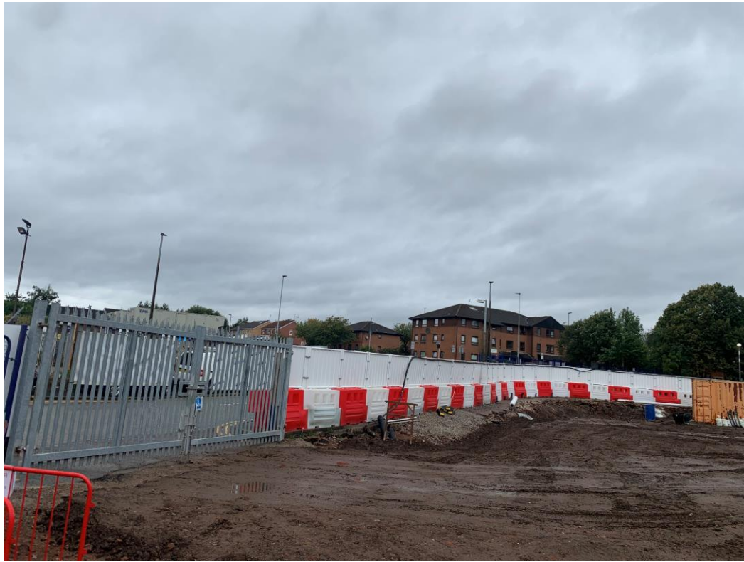
Site activity site formation piling mat
