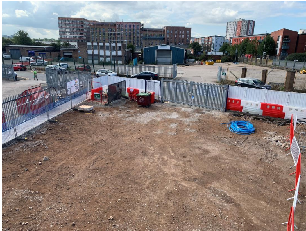
Site activity site formation levelling
