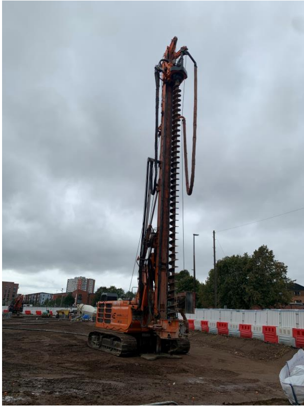
Auger piling rig
