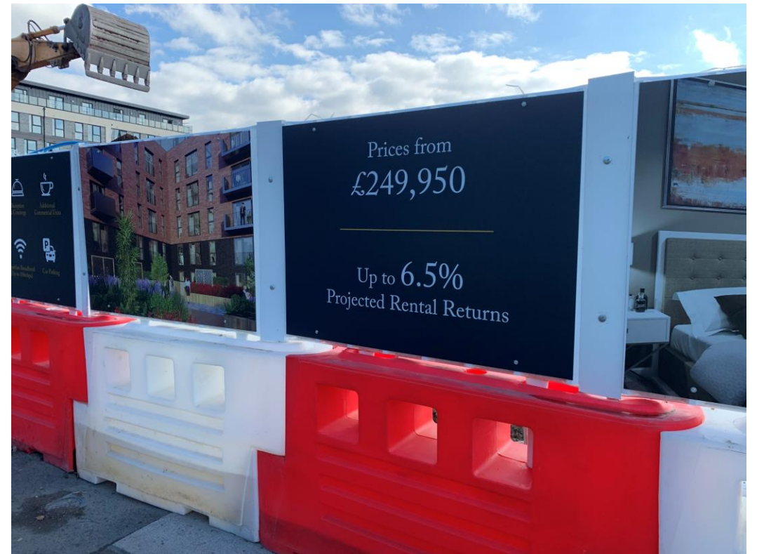
Ordsall Lane site view – site hoardings
