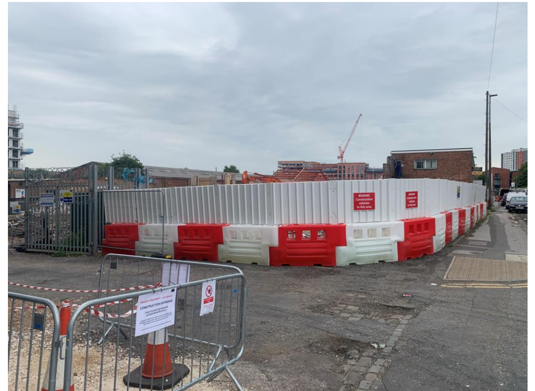
Ordsall Lane site view – buildings demolished
