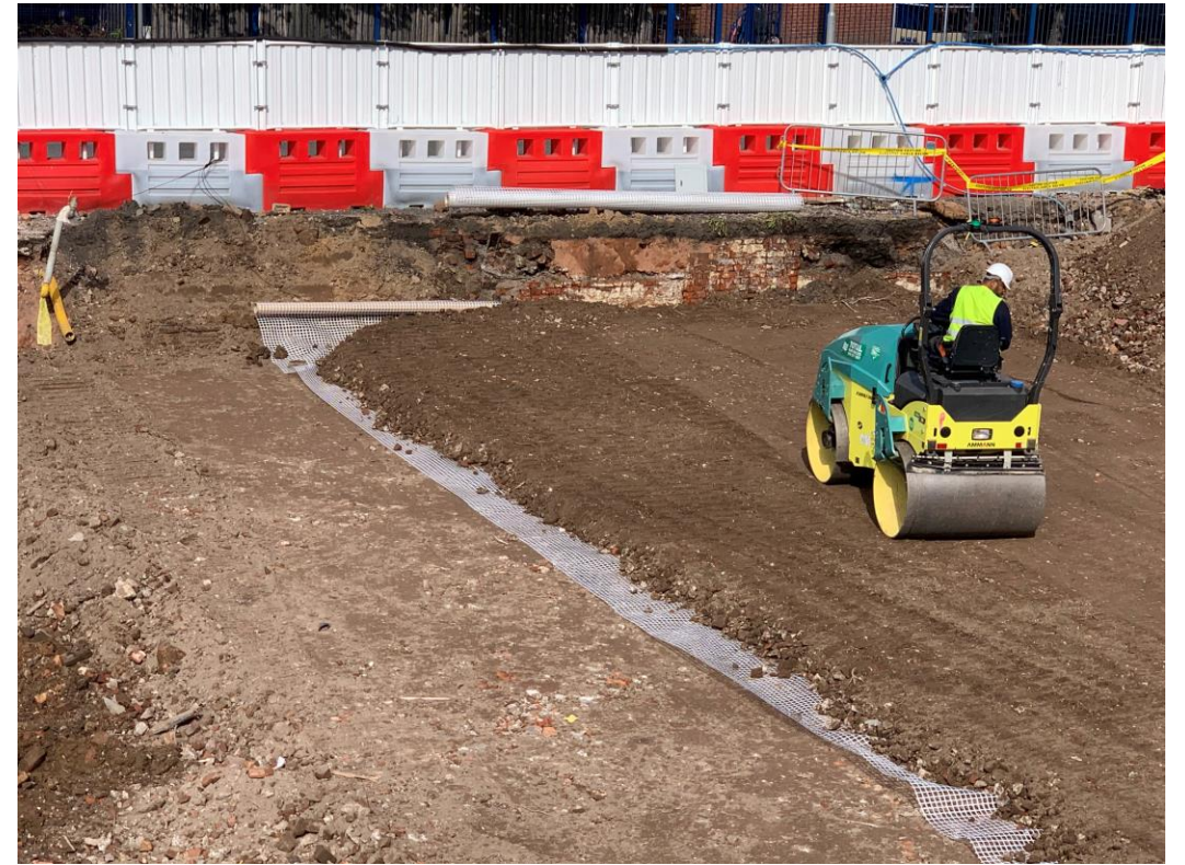
Site activity site formation levelling
