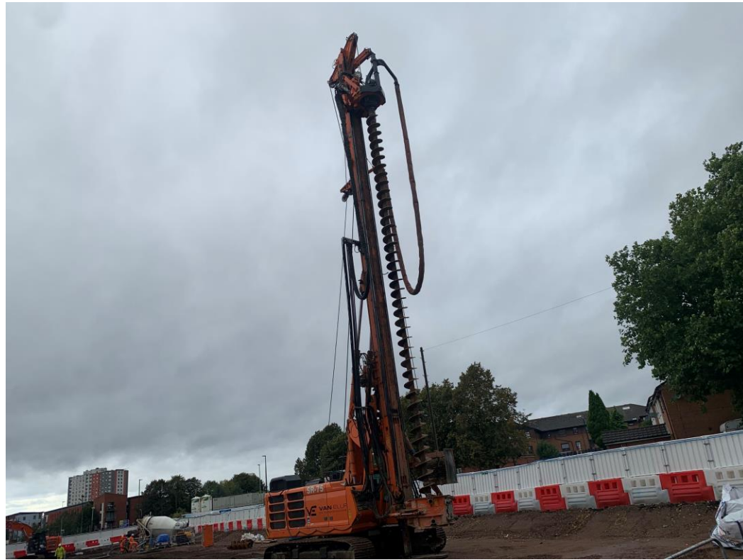
Auger piling rig
