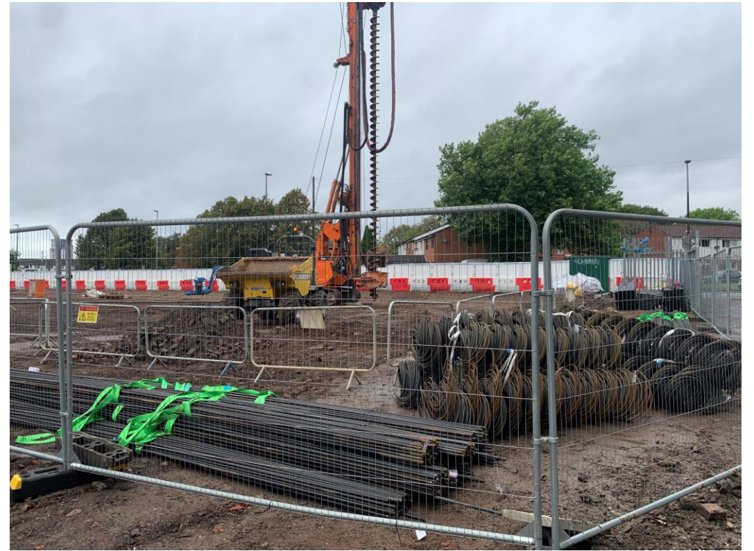
Piling cage reinforcement
