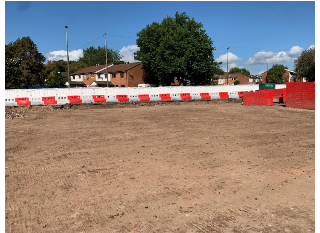
Site activity site formation levelling
