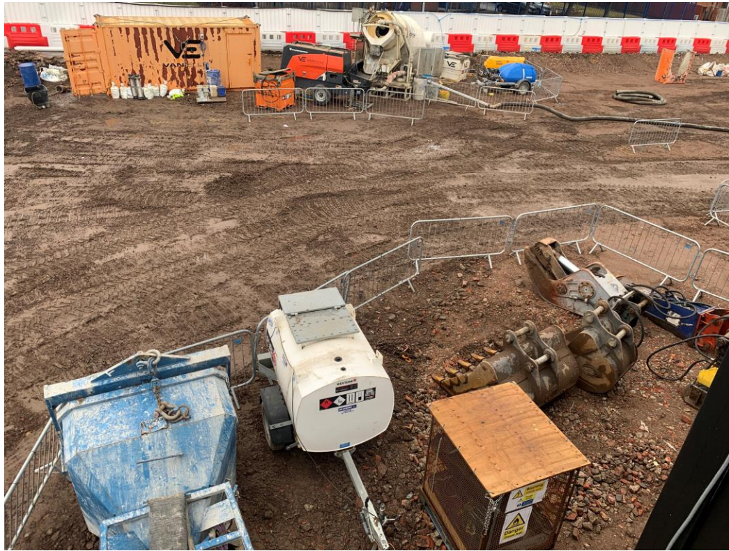
Site activity site formation piling mat
