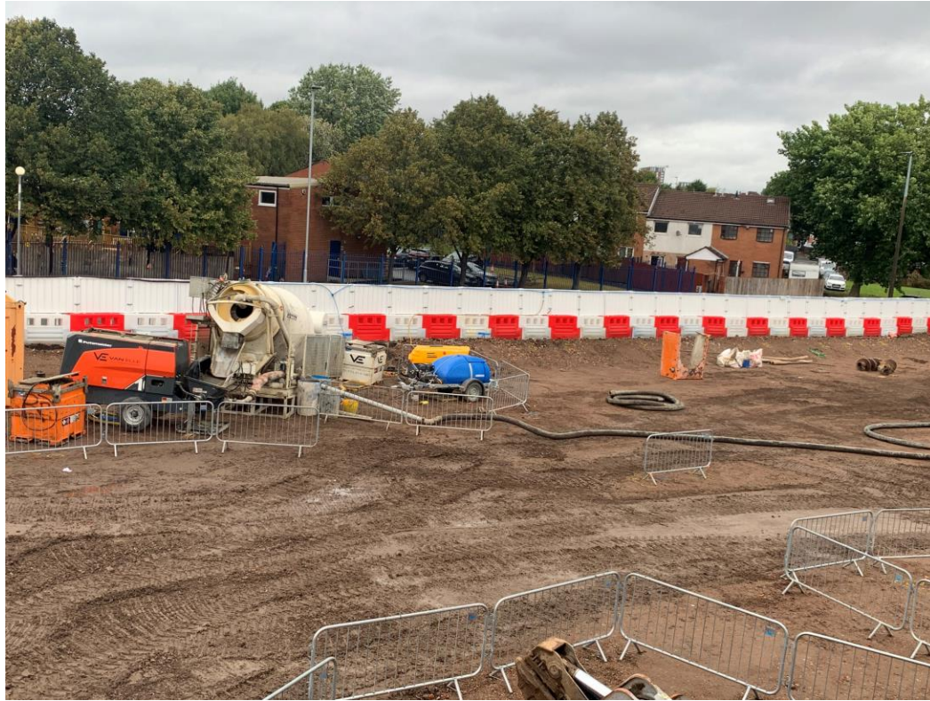
Site activity site formation piling mat
