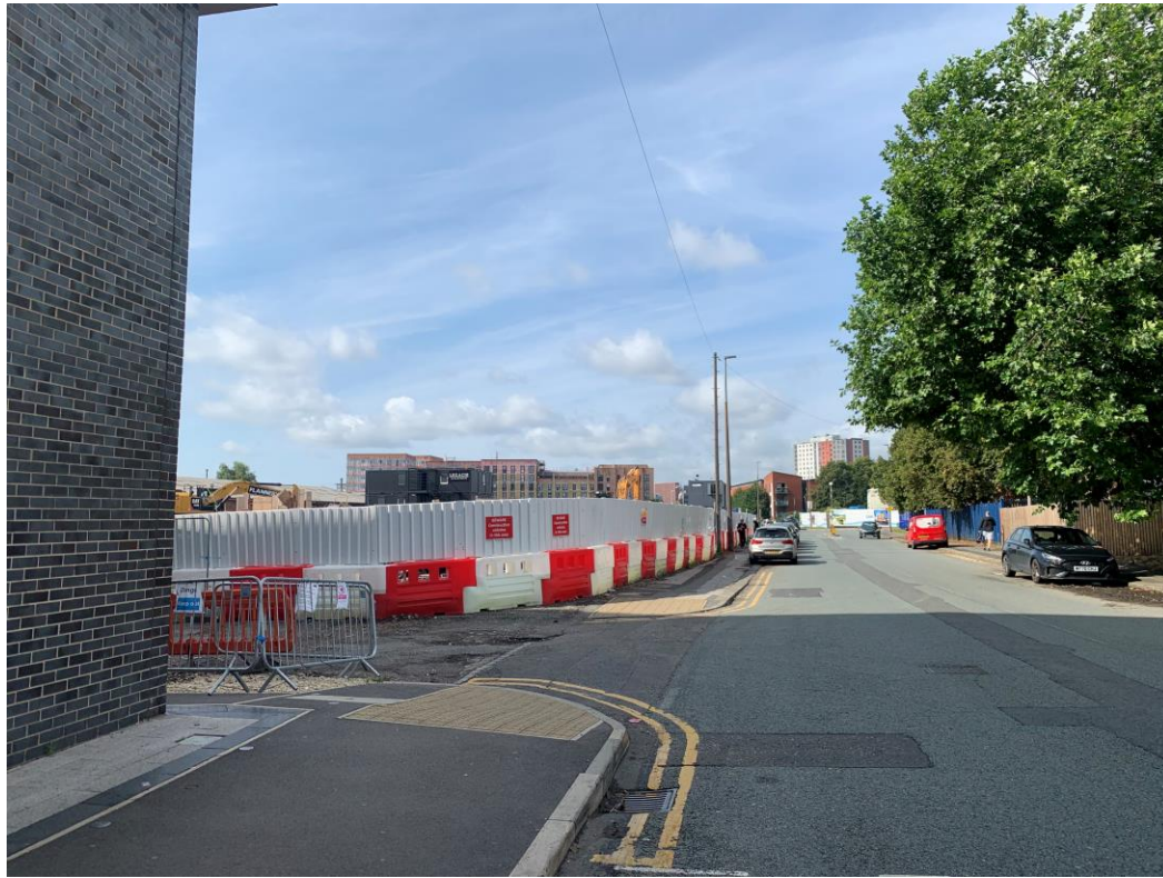
Ordsall Lane site view – buildings removed
