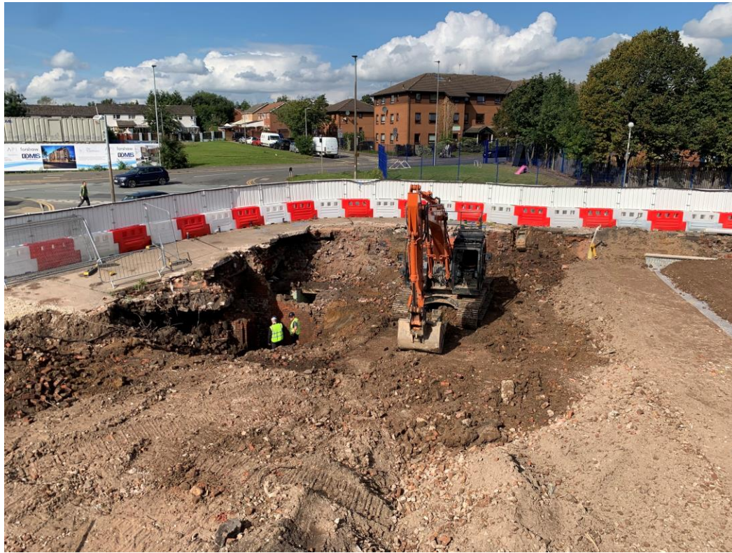
Site activity site formation levelling
