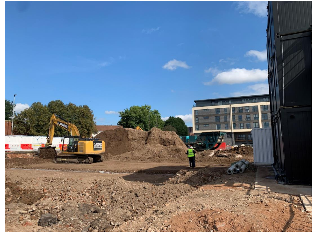
Site activity site levelling and stock piling
