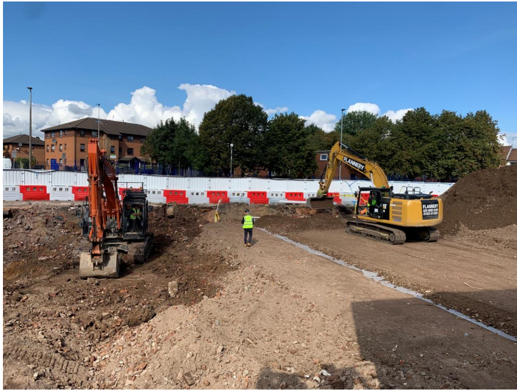
Site activity site levelling and stock piling
