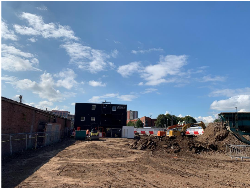
Site activity site levelling and stock piling
