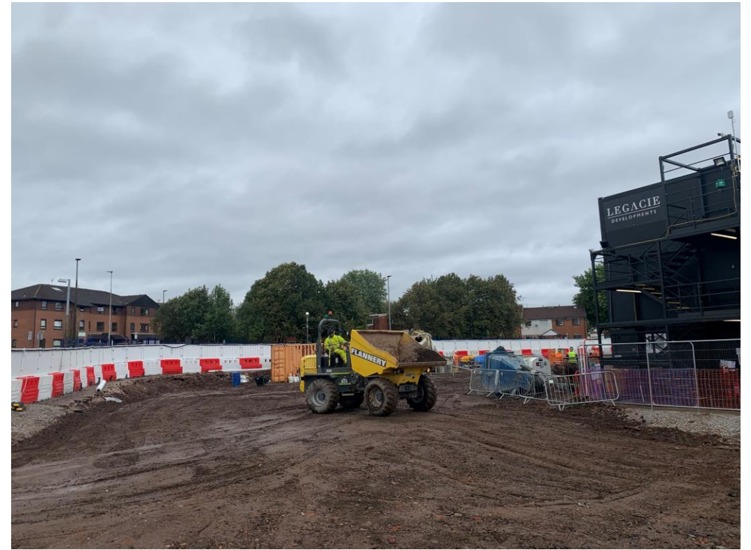
Site activity site formation piling mat
