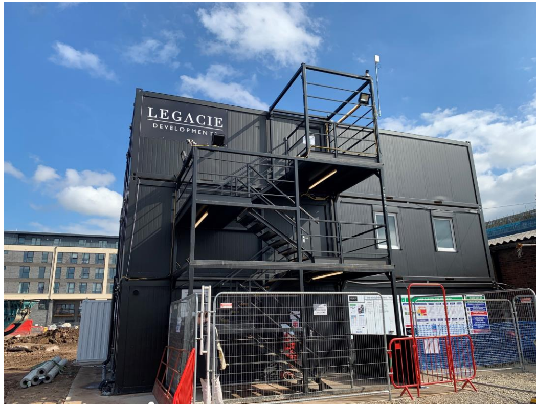
New site access & cabins
