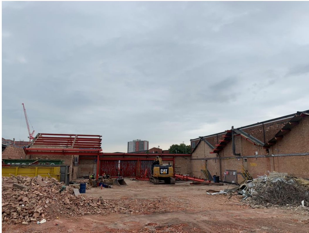
Site view – buildings demolished
