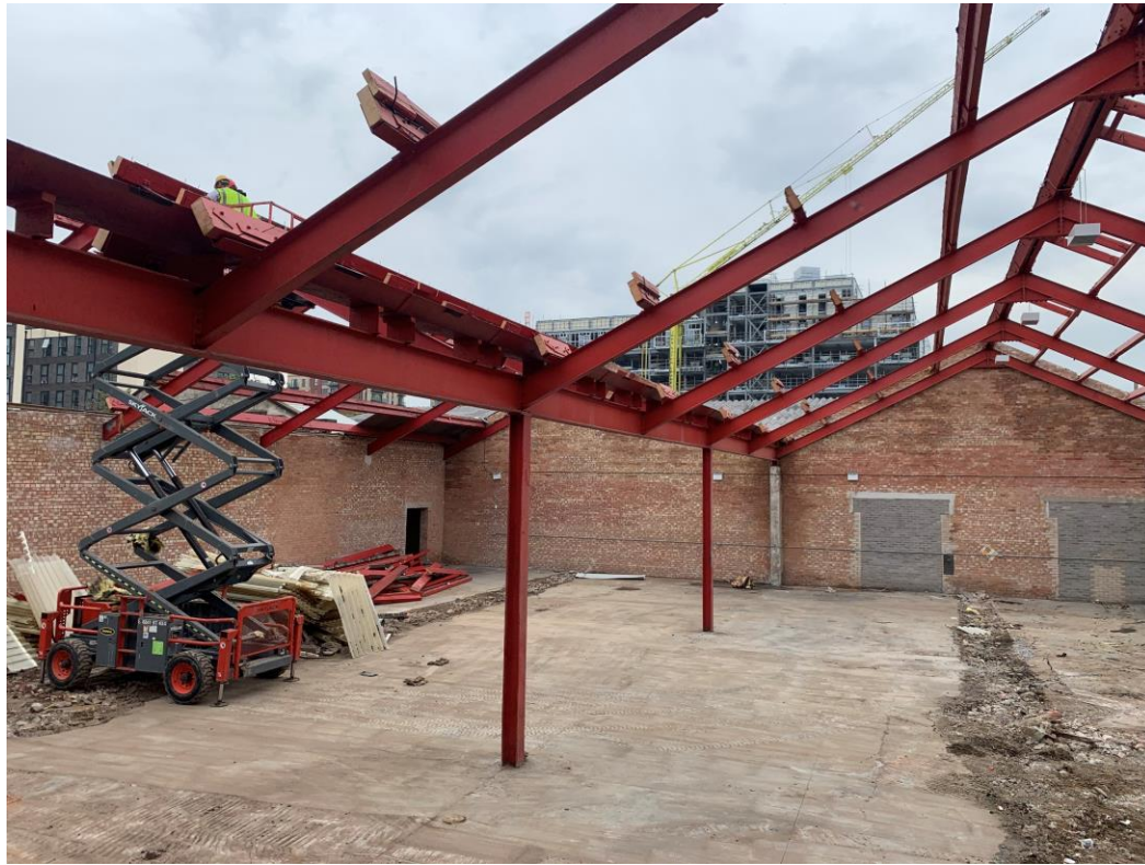
Building being demolished
