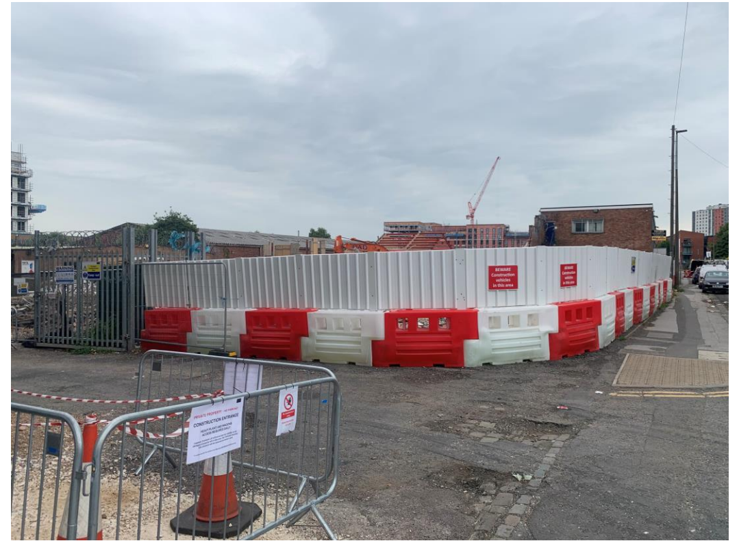
Ordsall Lane site view – buildings demolished
