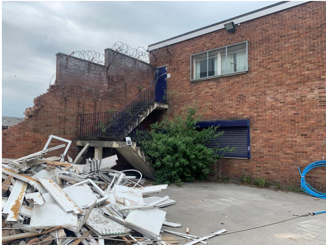
Site view – buildings demolished
