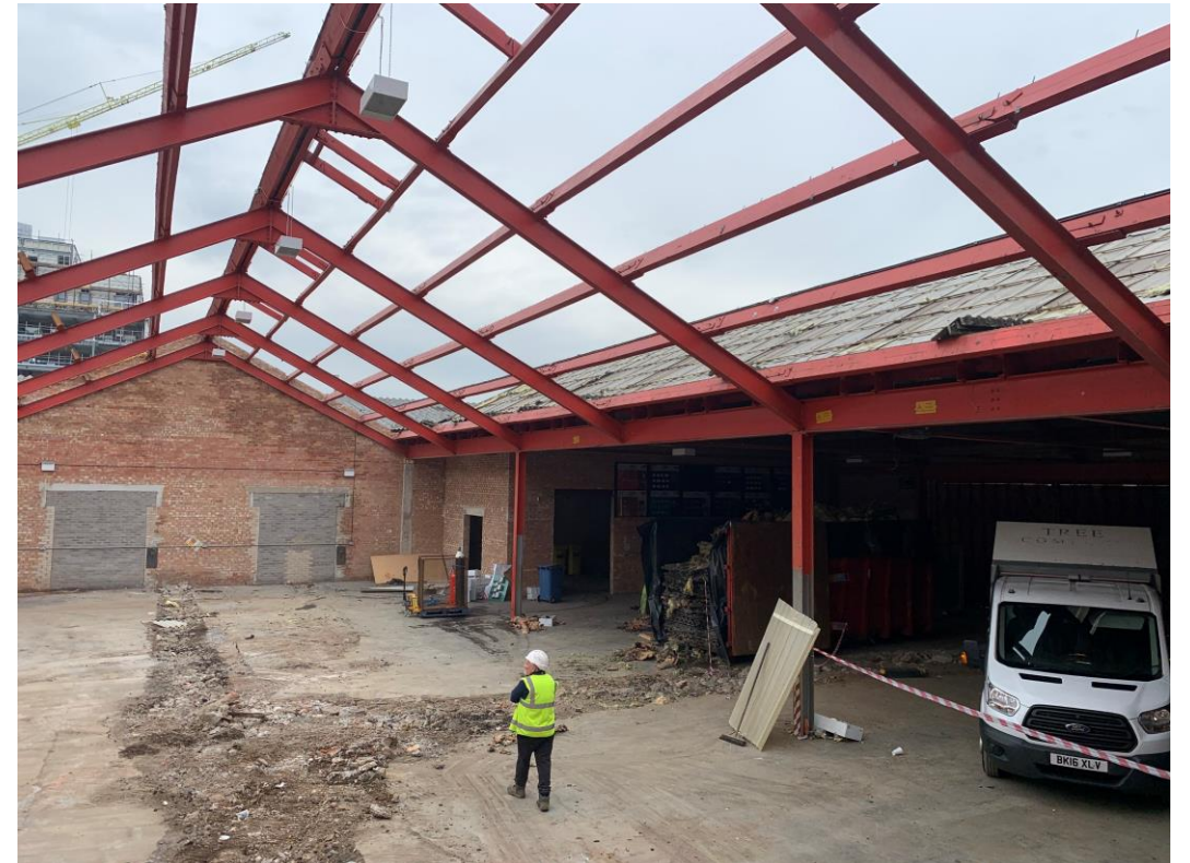
Building to be demolished
