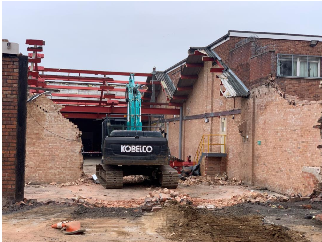
Building being demolished
