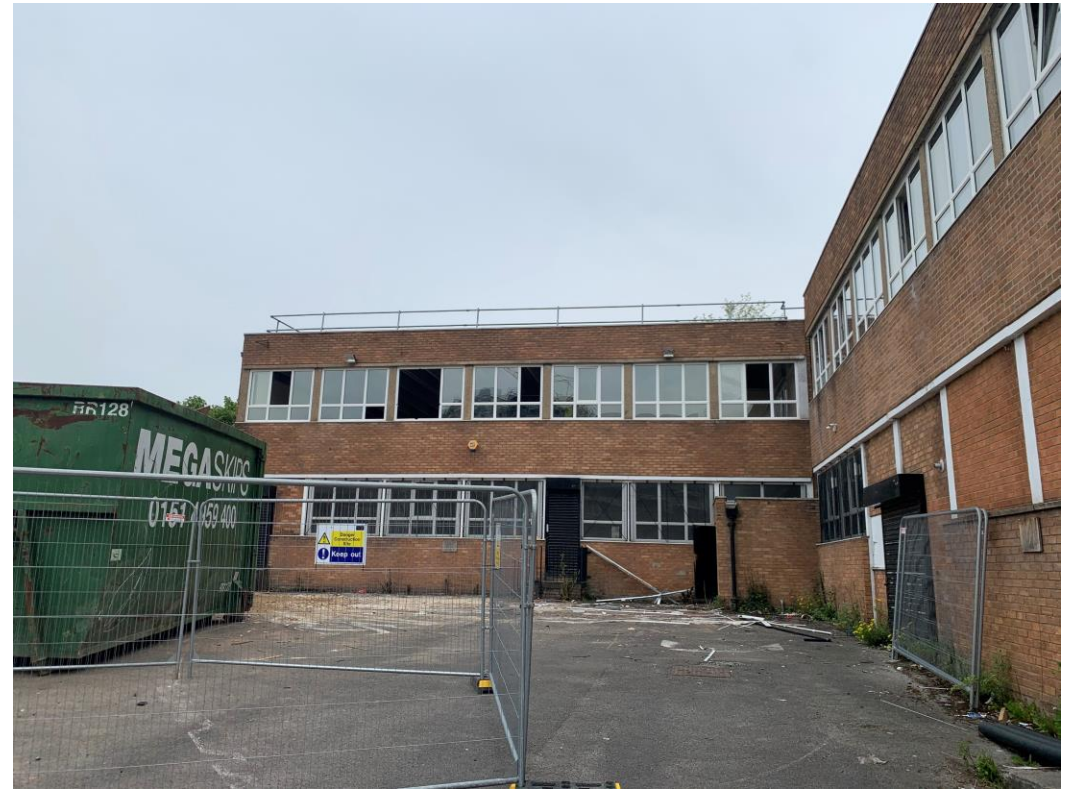
Dyer Street site view – buildings to be demolished
