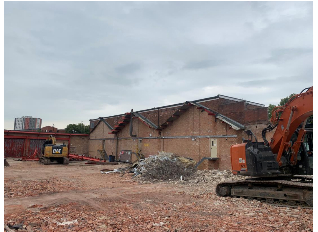
Site view – buildings demolished
