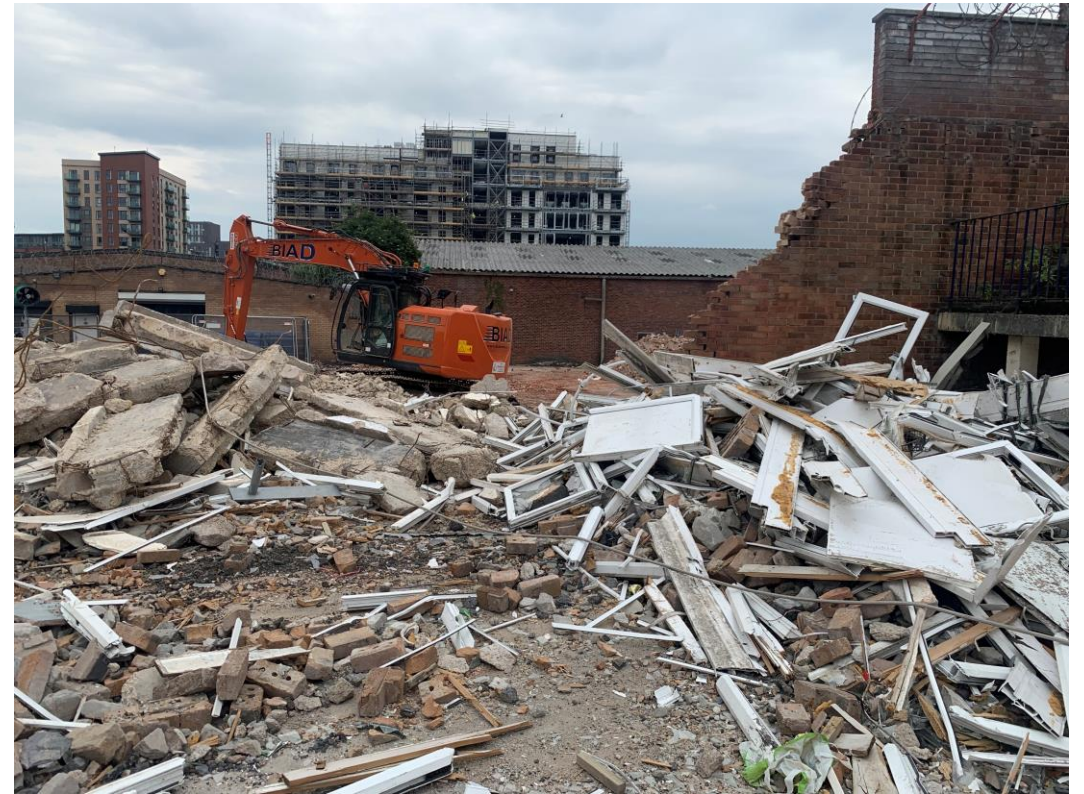
Site view – buildings demolished
