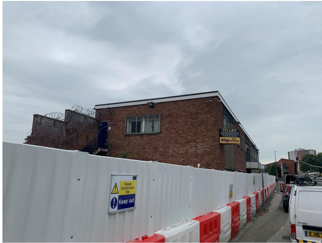
Ordsall Lane site view – buildings demolished
