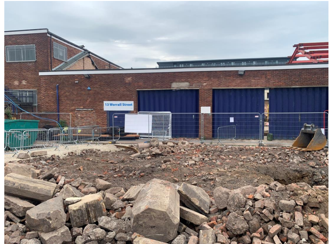
Site view – buildings to be demolished
