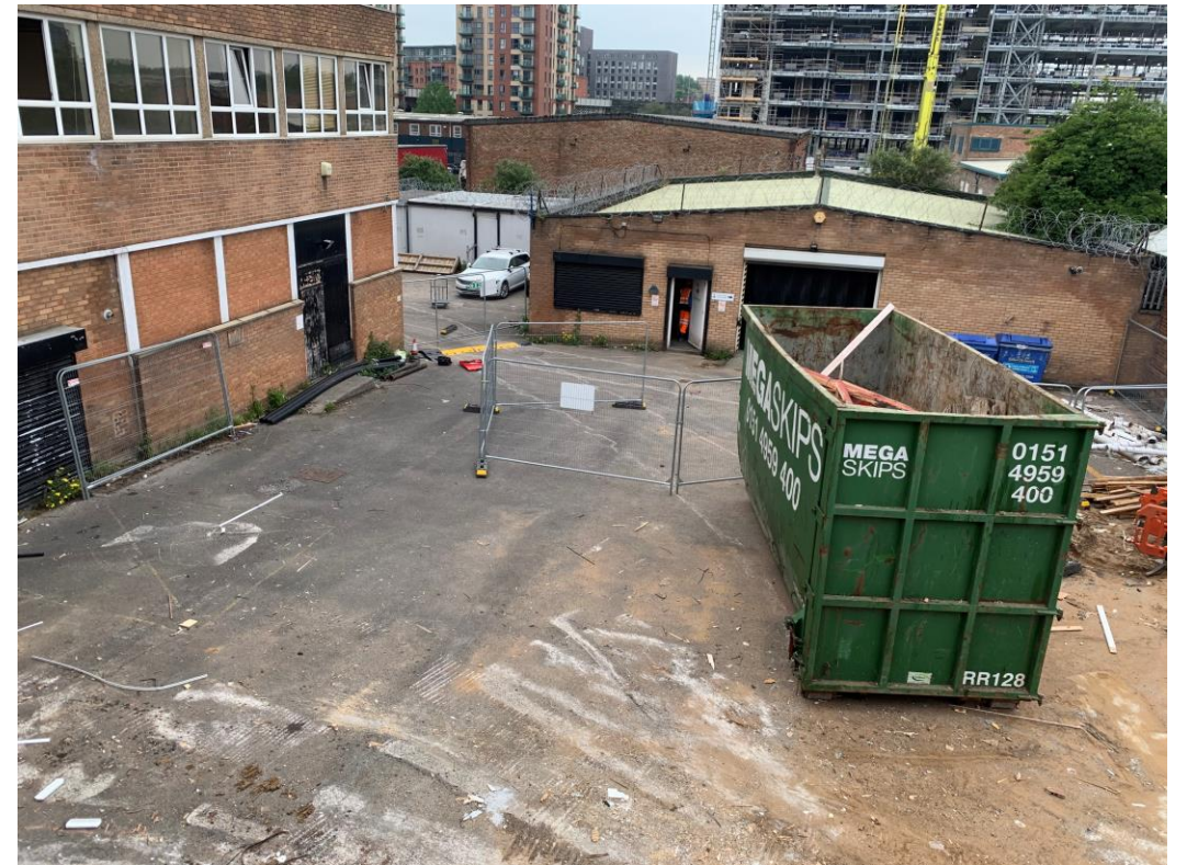
Building to be demolished
