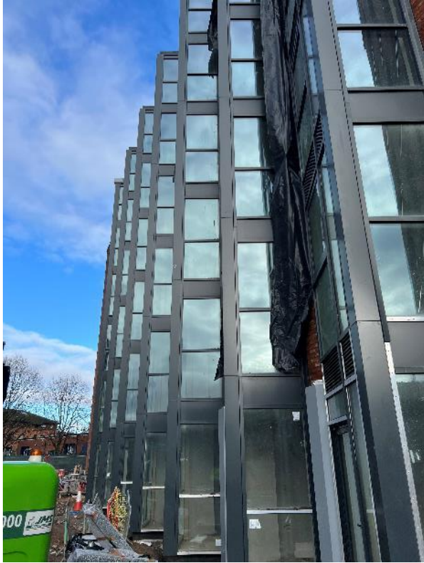
Block A - window and glazing panels
