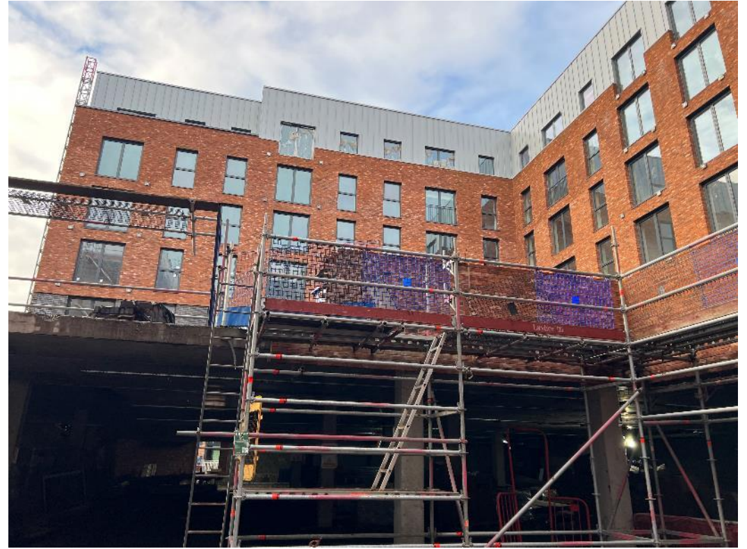
Podium site view
