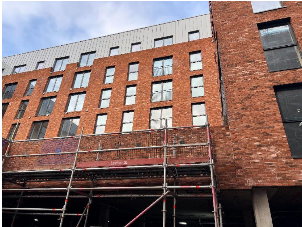
Podium site view
