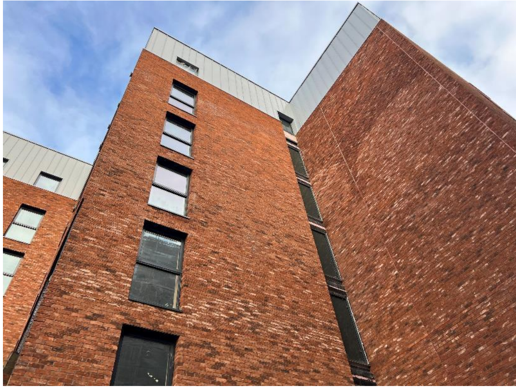
Podium site view
