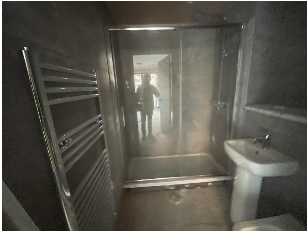
Level 2 – Shower screen installed
