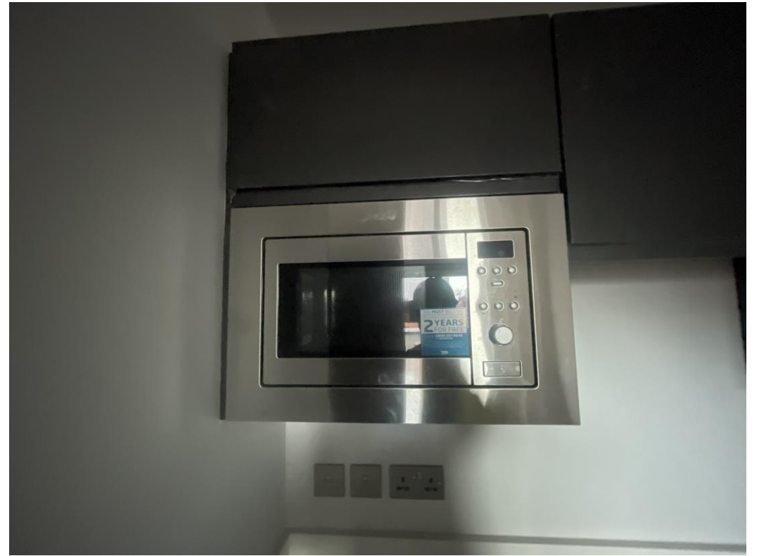
Level 6 – Kitchen appliances installed
