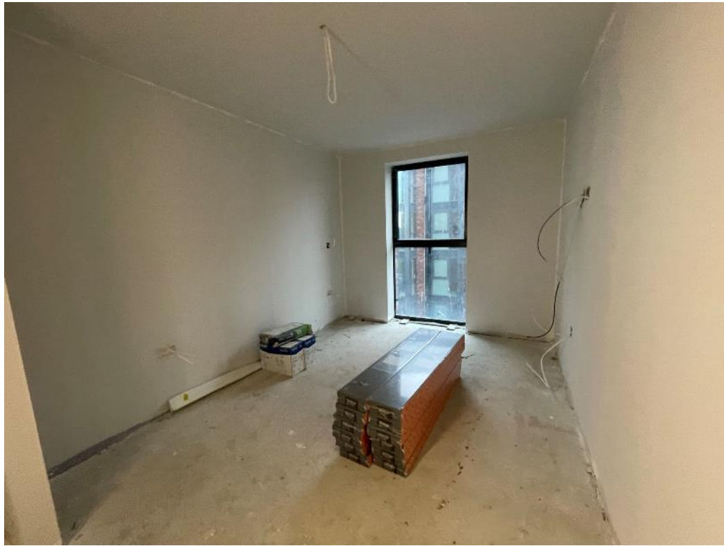
Level 6 – Hoist apartment wall & ceiling decoration
