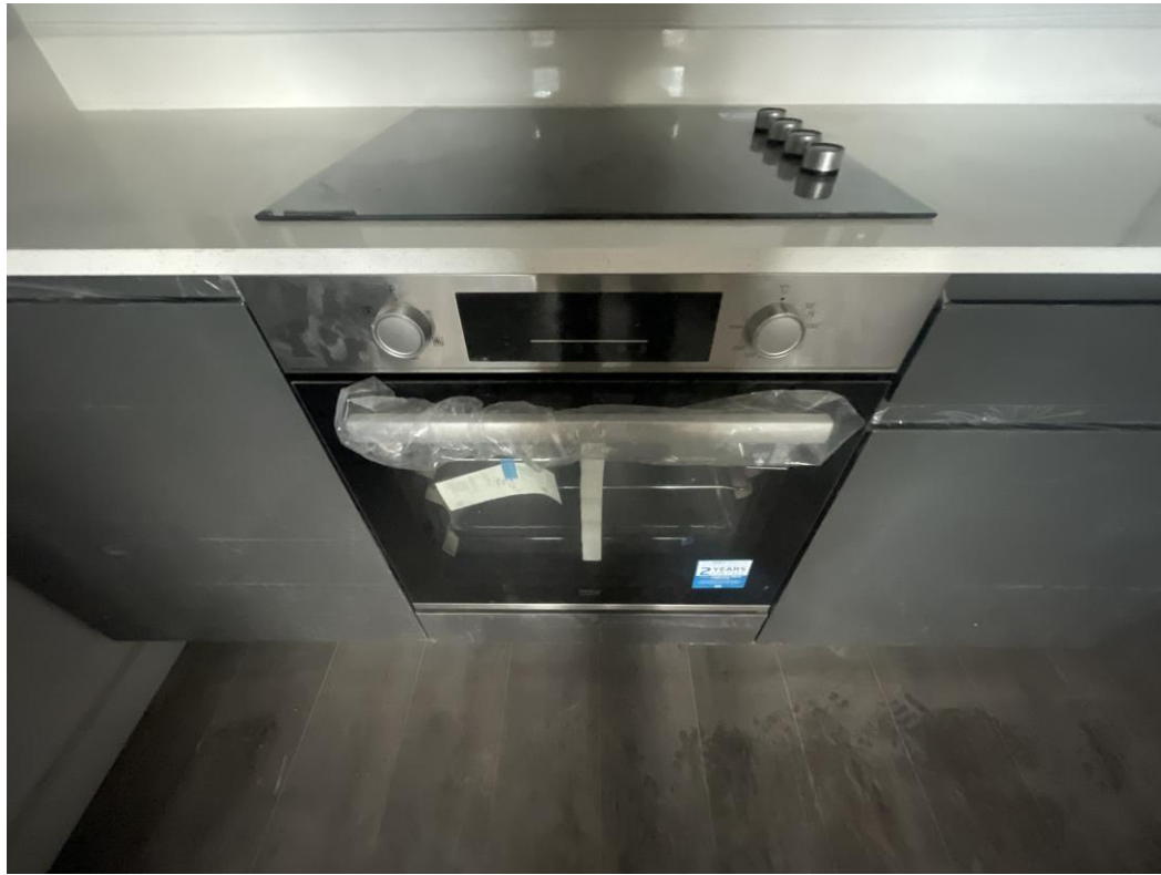
Level 6 – Kitchen appliances installed
