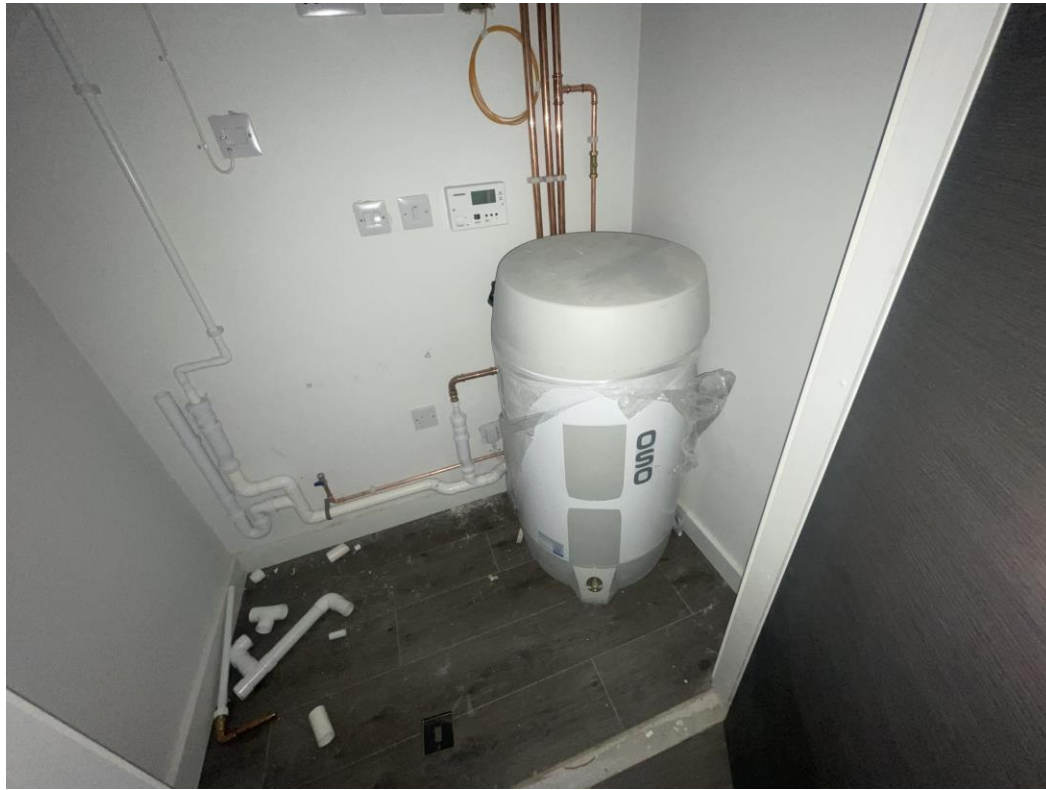
Level 6 – Second fix mechanical appliances
