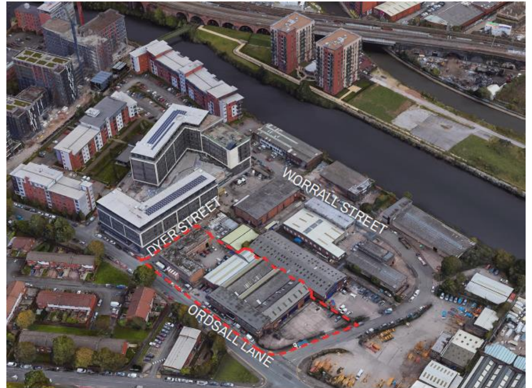
Aerial view of Merchant's Wharf site location
