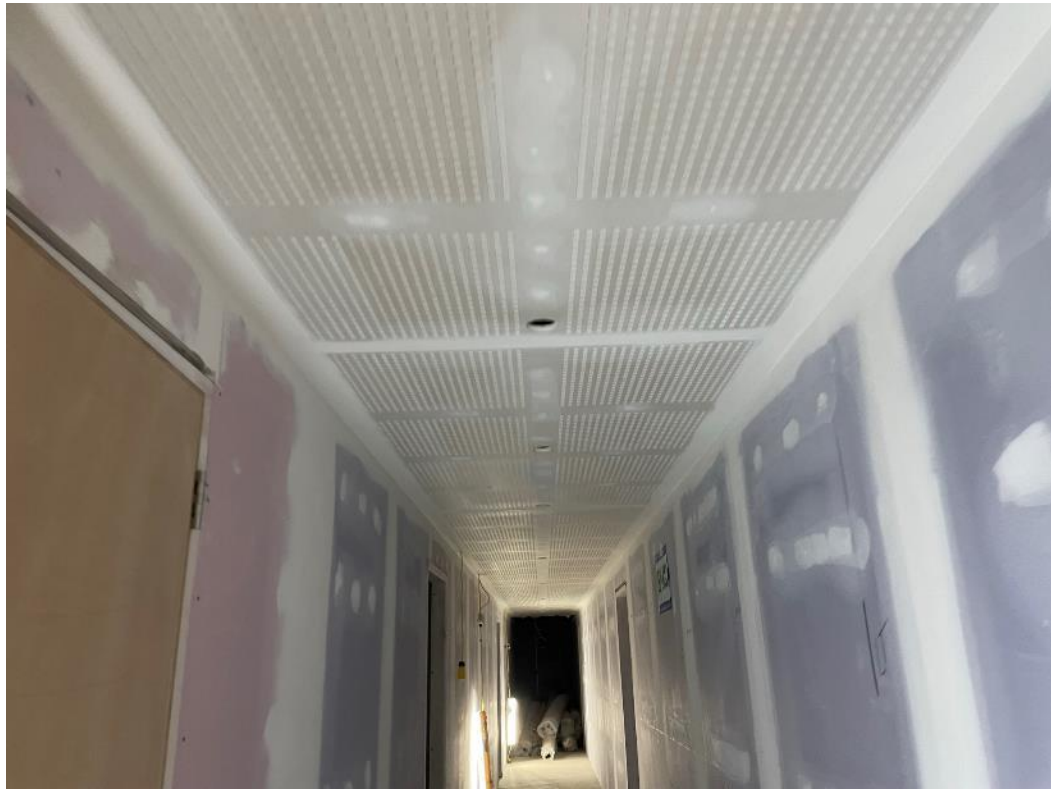
Level 3 – Acoustic ceiling decoration corridor
