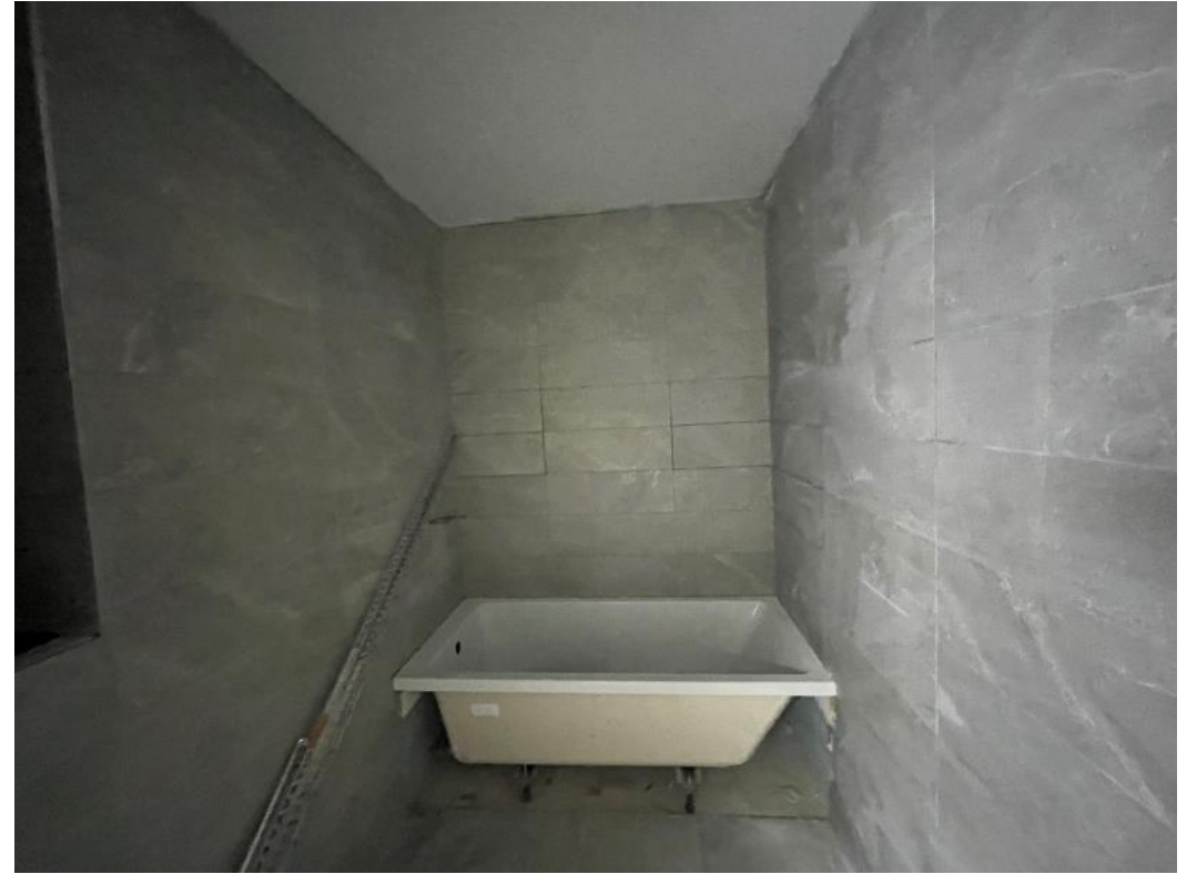
Level 4 – Bathroom wall & floor tiling
