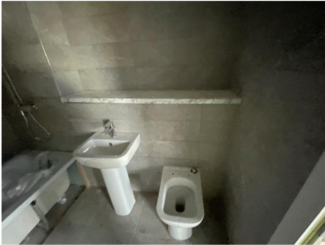
Level 8 – Bathroom sanitary appliances
