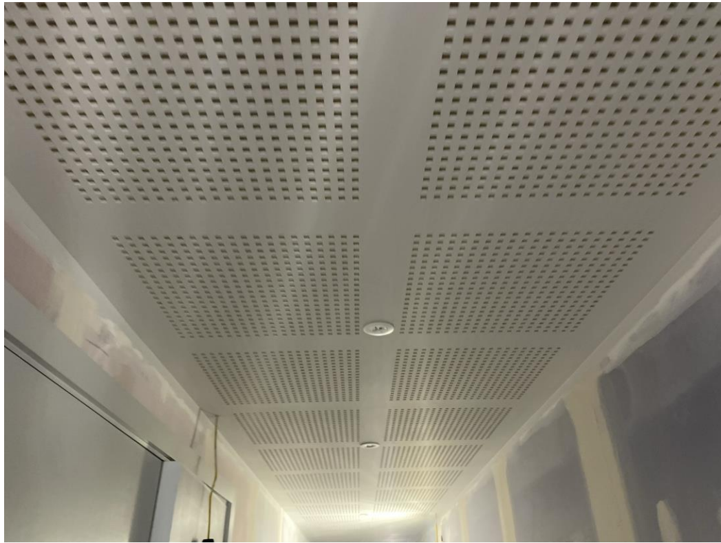
Level 5 – Acoustic ceiling decoration corridor
