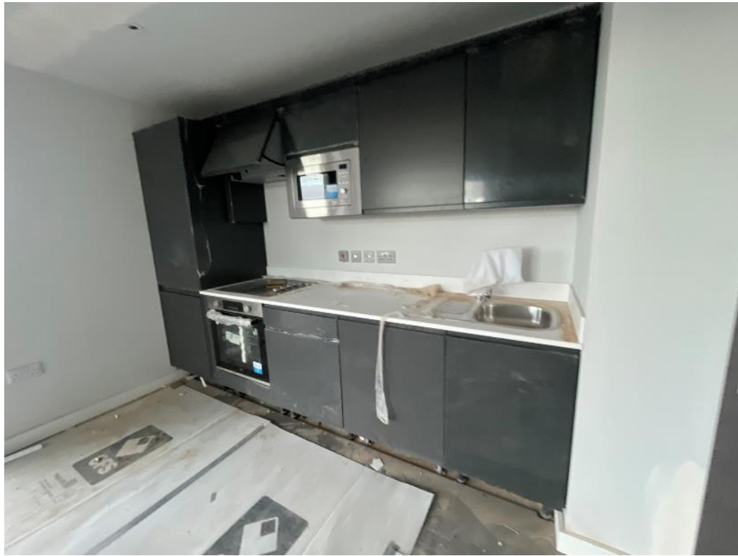
Level 5 – Kitchen complete
