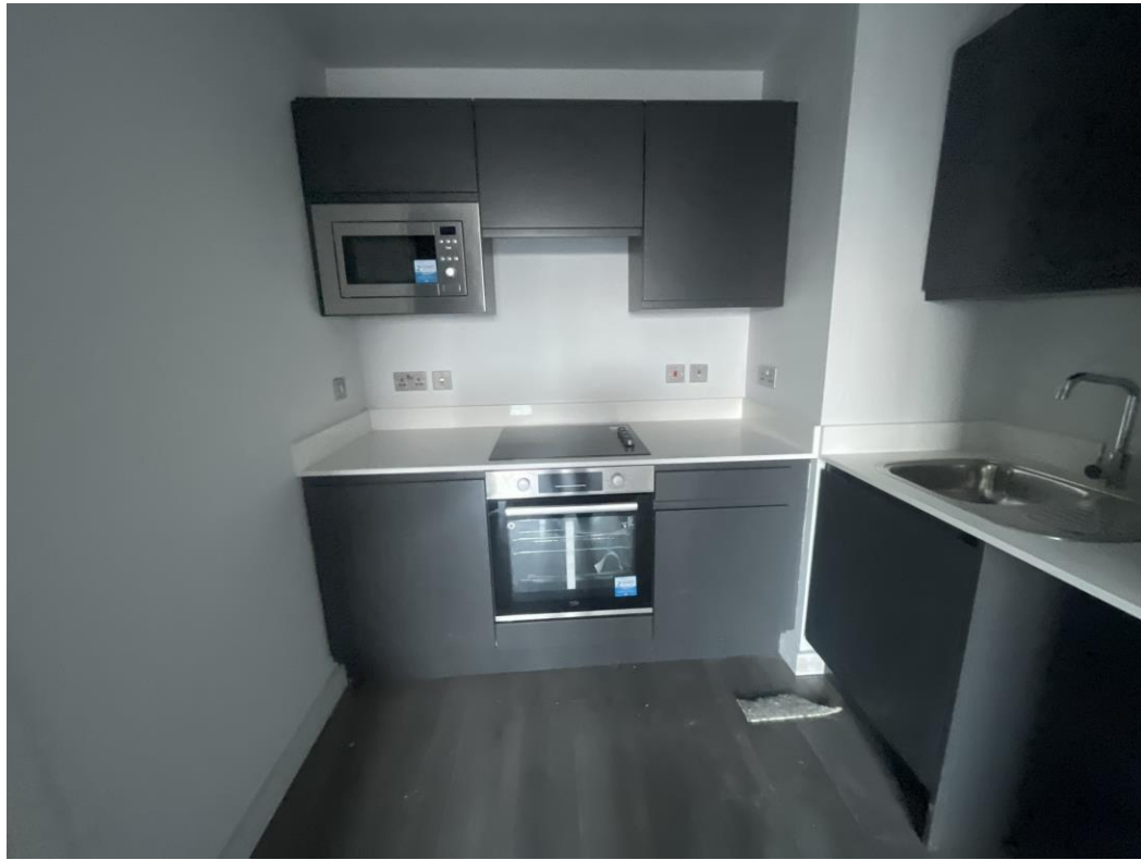
Level 5 – Kitchen units installed
