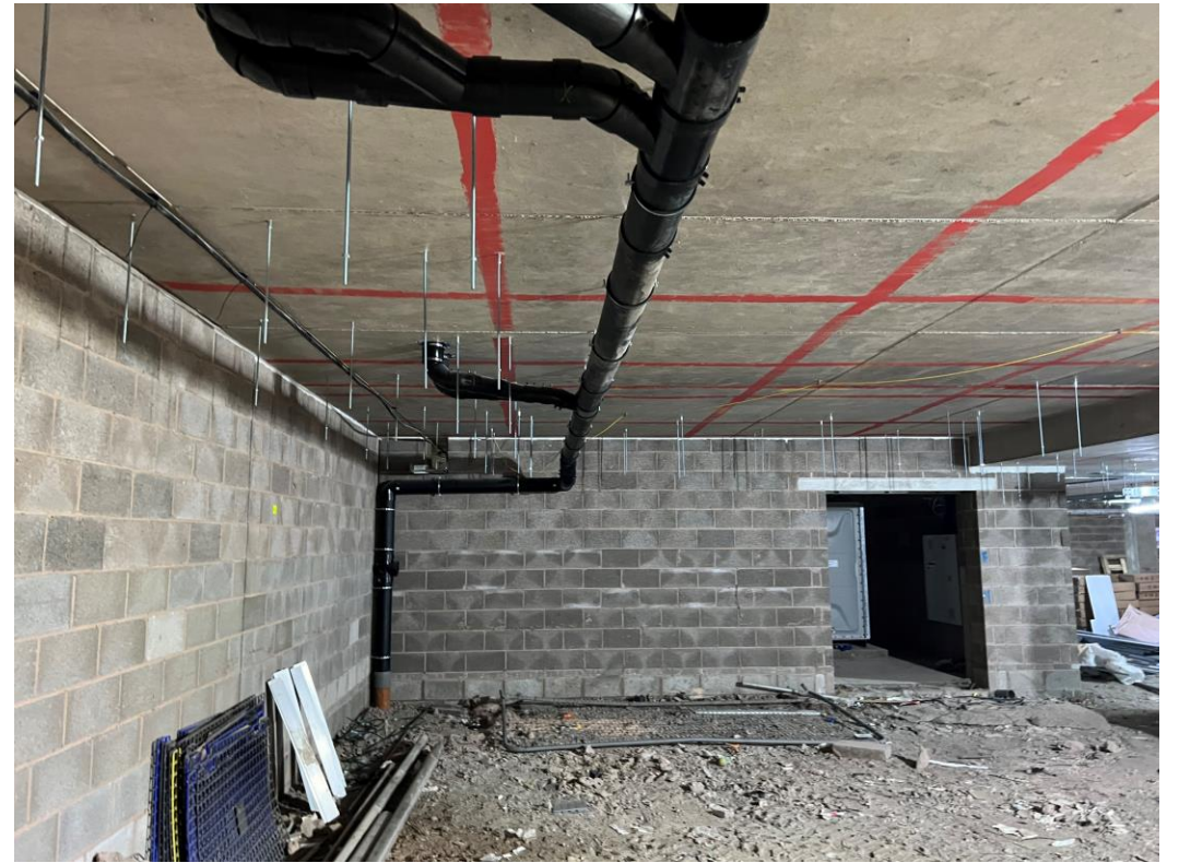
Ground Floor – 1 st Fix M&E
