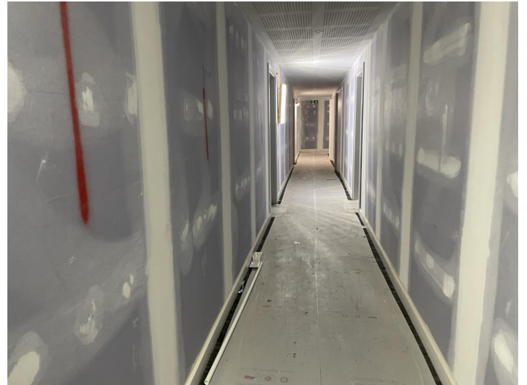
Level 1 – Wall tape & jointing
