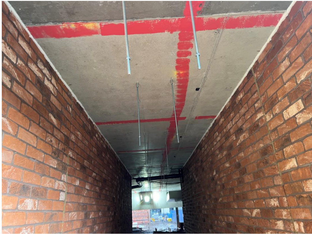
Ground Floor – Fixing rods in place for cable trays
