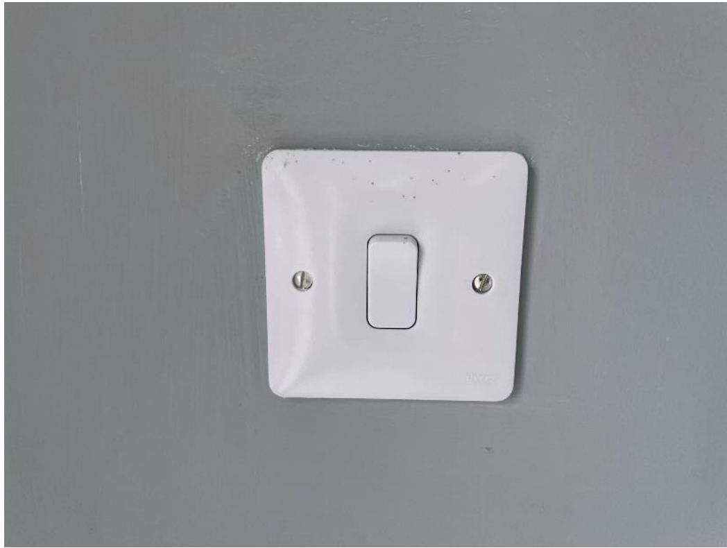
Level 1 – 2 nd fix electrical
