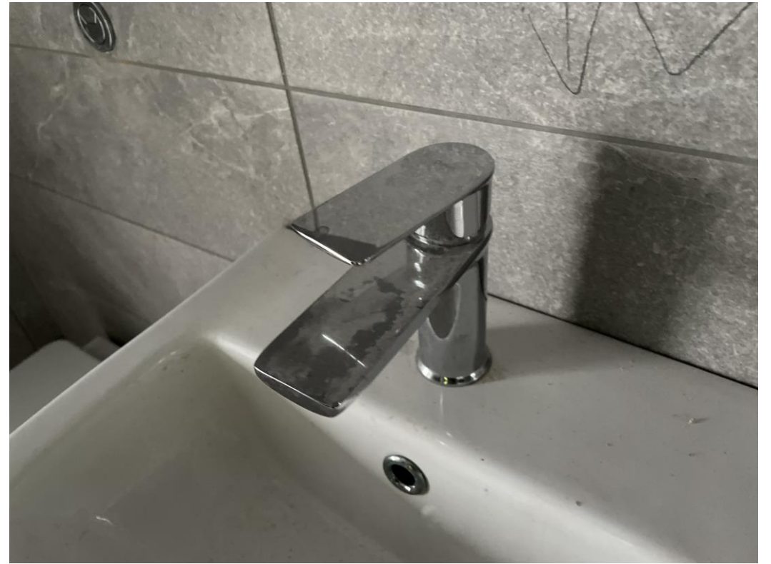
Level 6 – WHB taps installed
