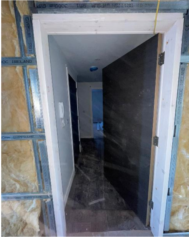
Level 2 – Hoist apartment doors installed
