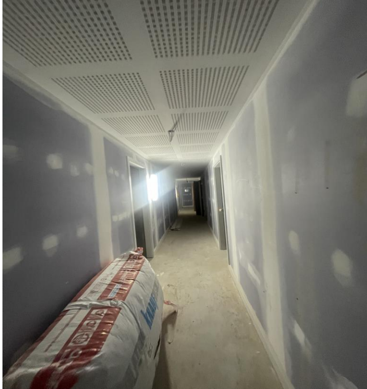
Level 1 – Acoustic ceiling decoration corridor
