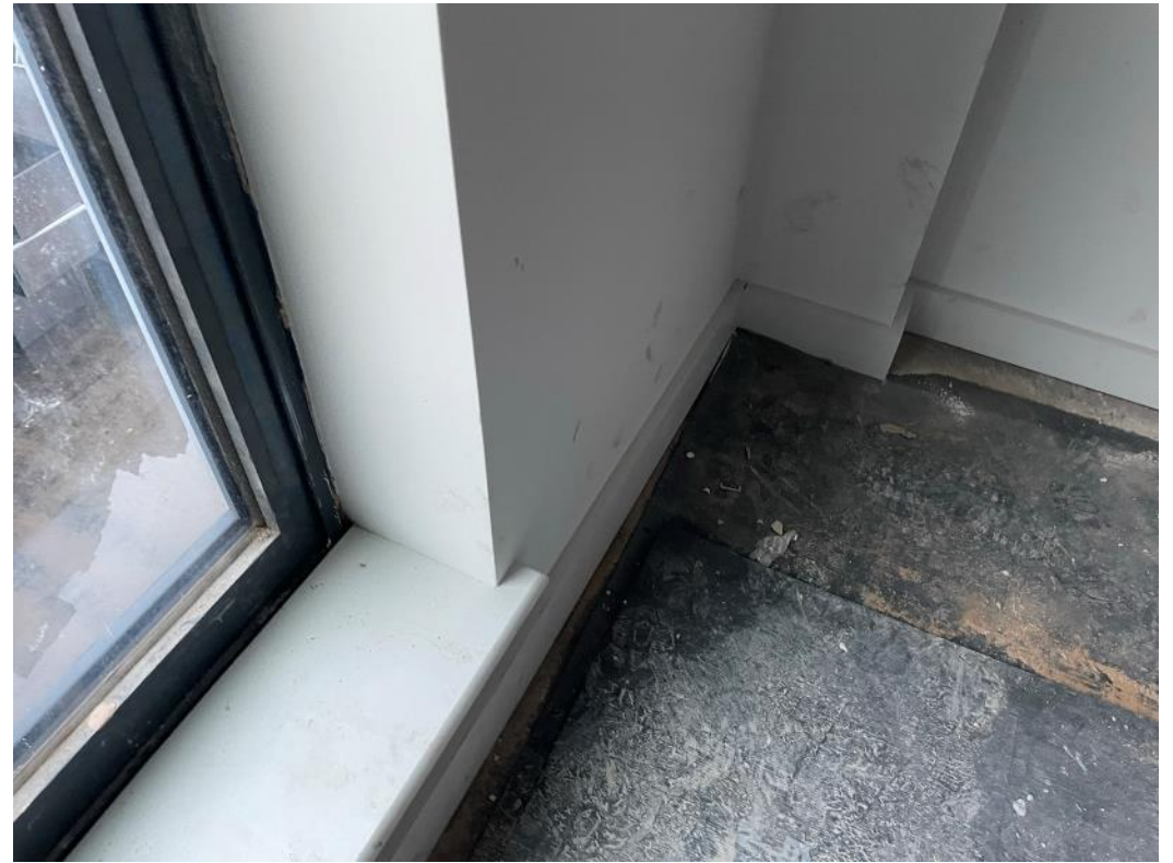
Level 7 – 2 nd fix joinery
