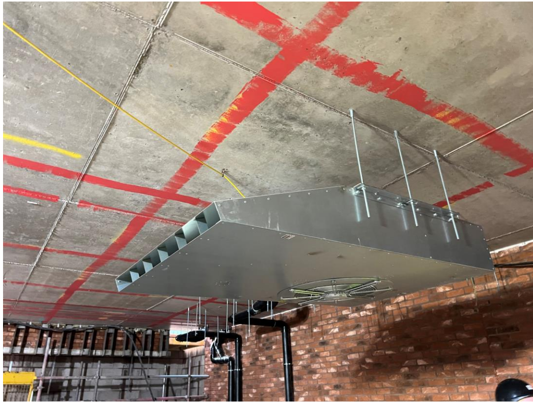
Ground Floor – 1 st Fix M&E
