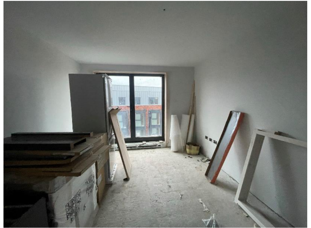
Level 6 – Hoist apartment wall & ceiling decoration
