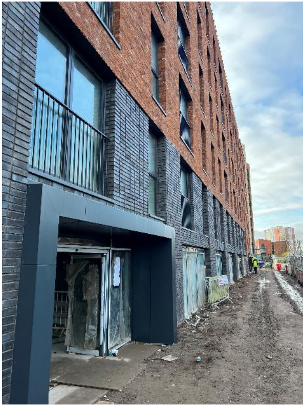
Cladding installed to entrance canopy
