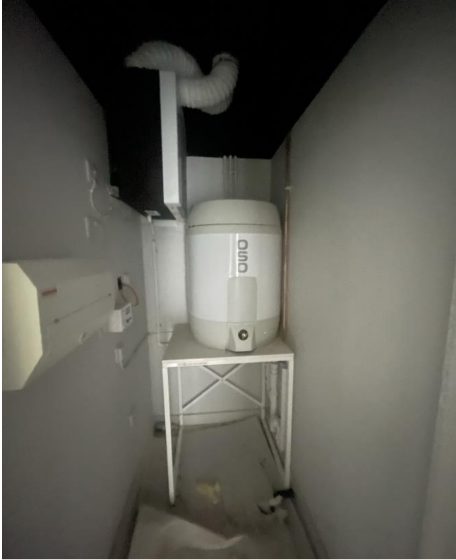
Level 3 – 2 nd fix mechanical & electrical
