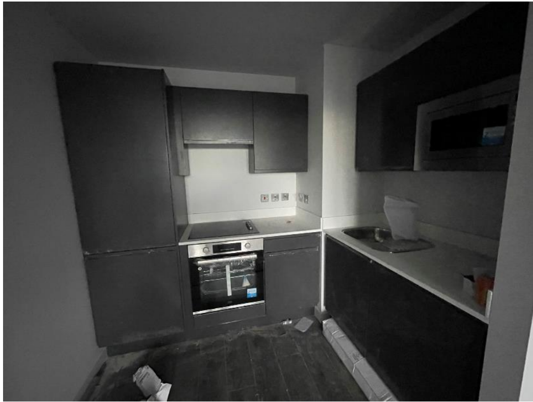
Level 6 – Kitchen units & worktops installed
