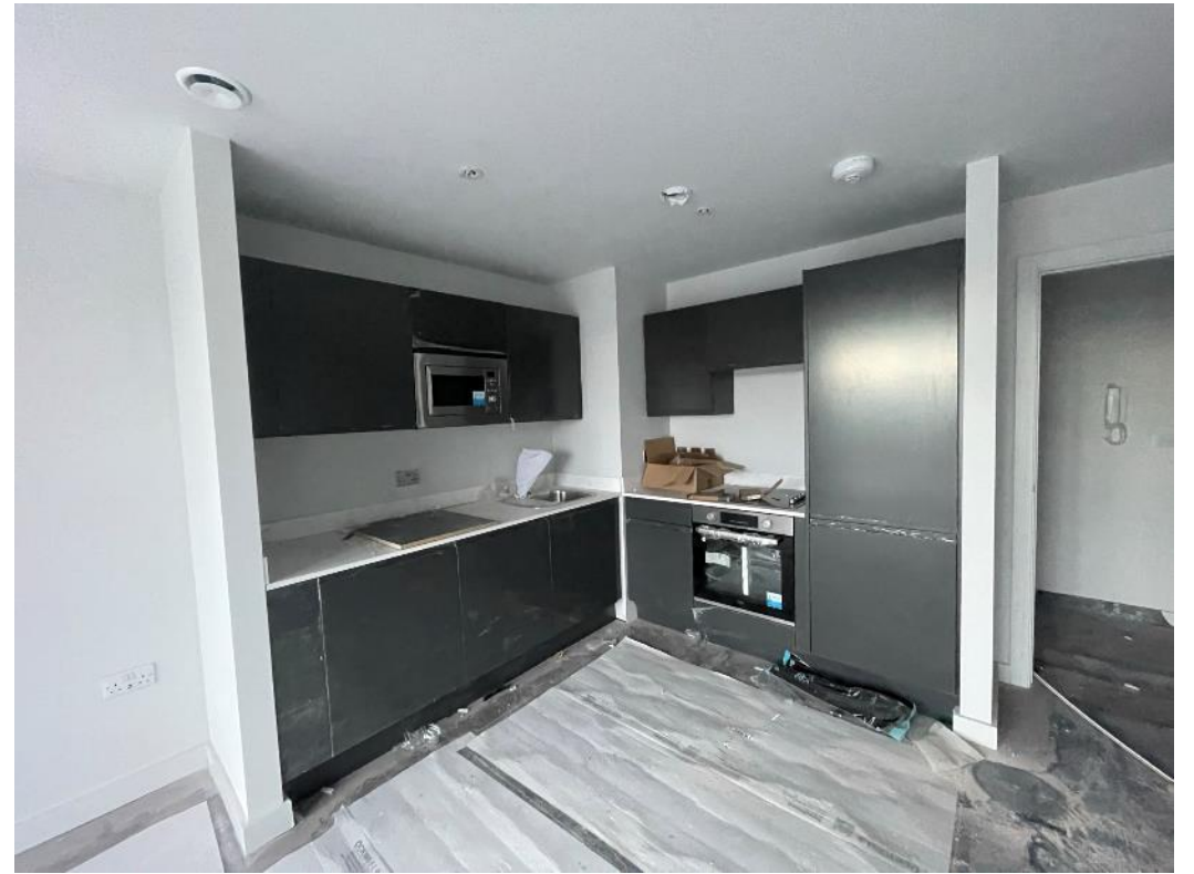
Level 6 – Kitchen units & worktops installed
