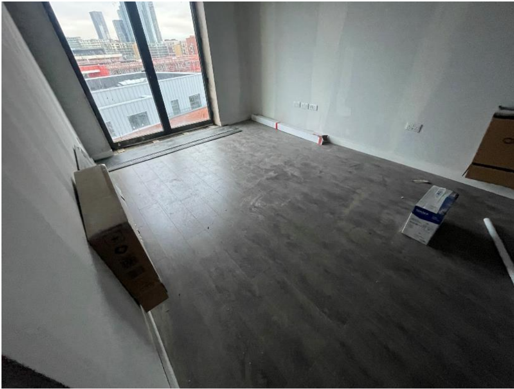
Level 8 – Laminate flooring installed
