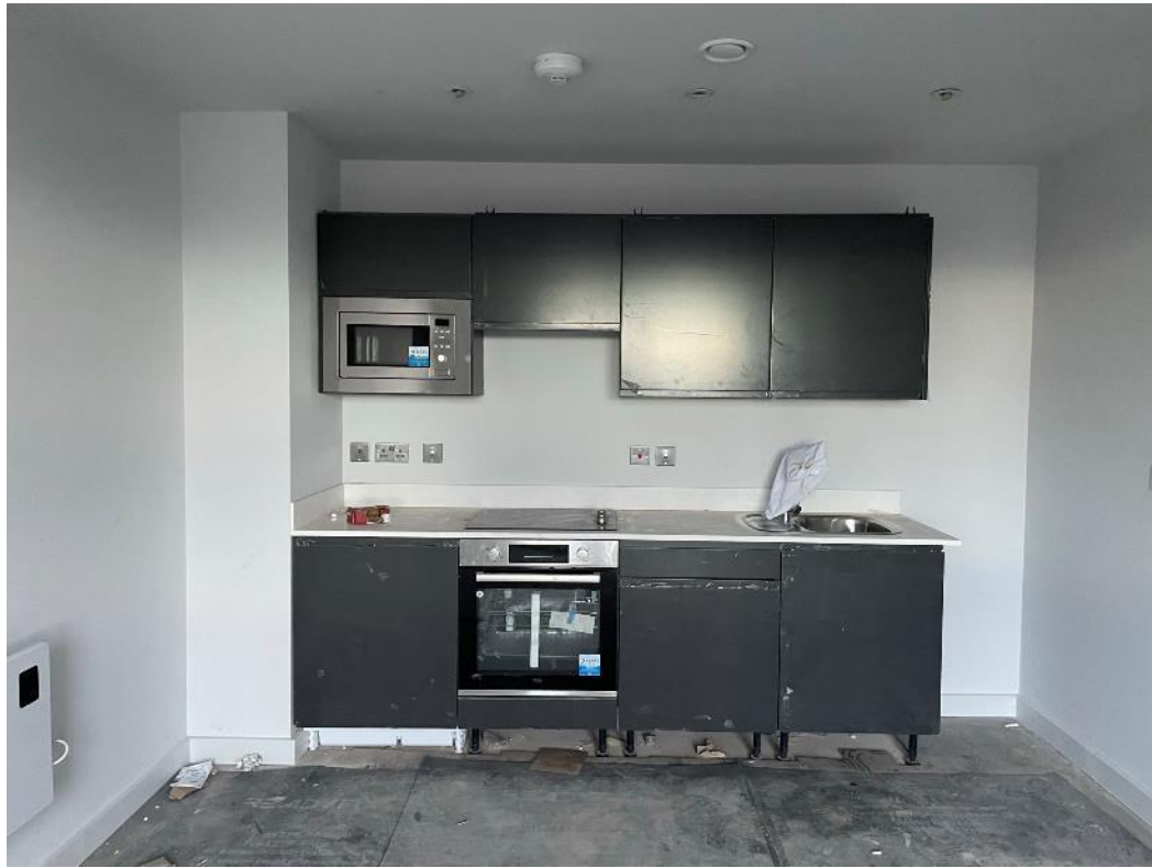
Level 8 – Kitchen units & worktops installed
