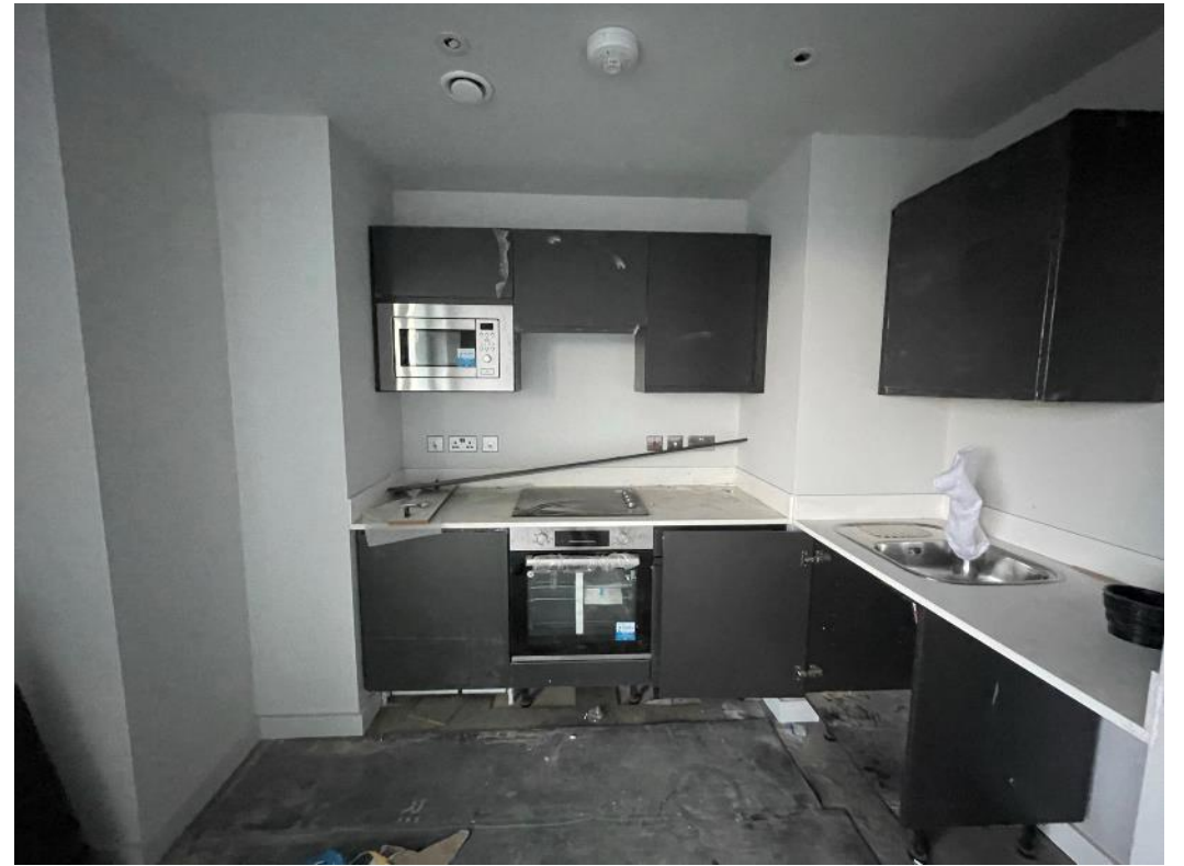
Level 8 – kitchen installed
