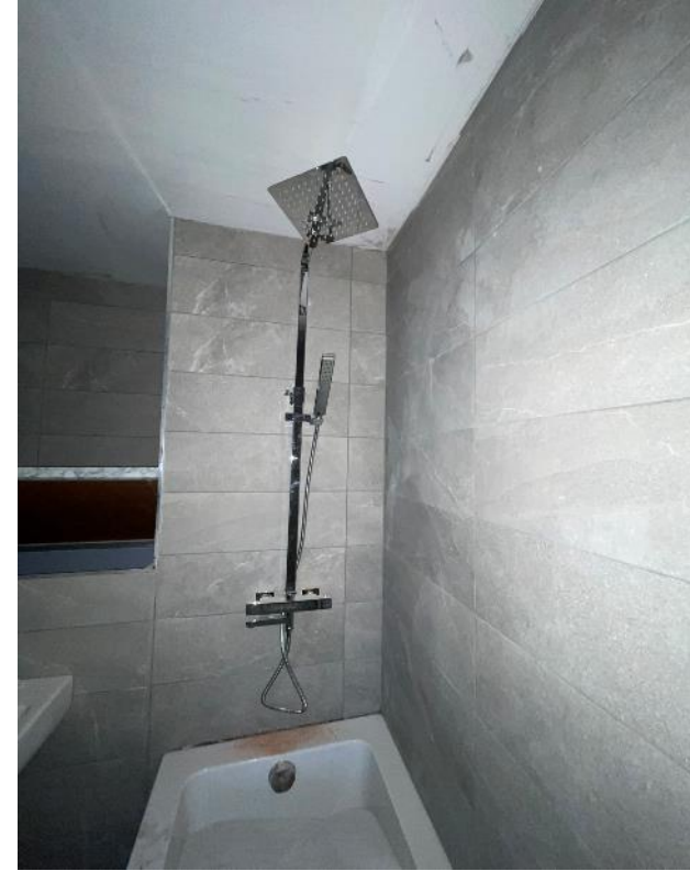
Level 5 – Shower bar installed
