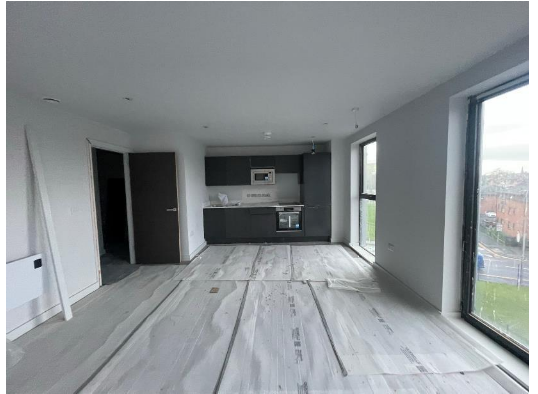
Level 5 – Kitchen complete
