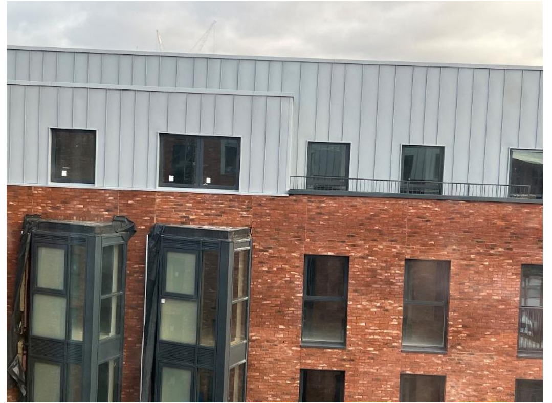
Block B parapet handrails
