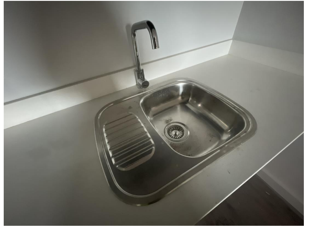
Level 6 – Kitchen sink and tap
