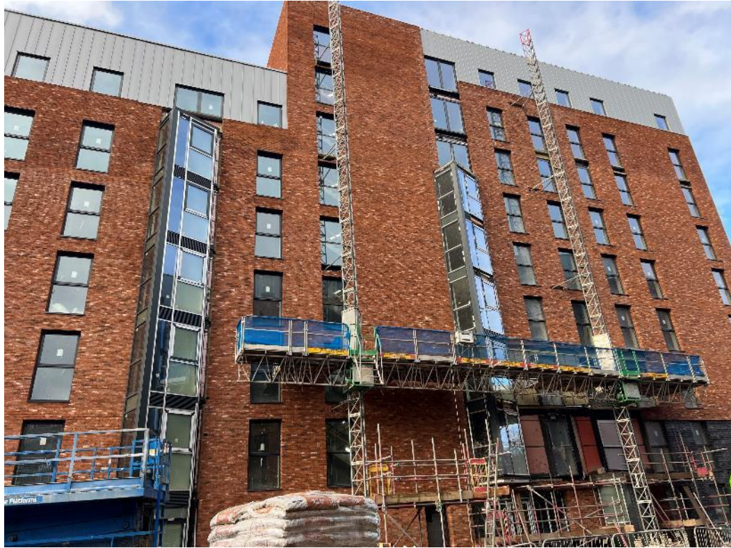
Block B wall insulation and cladding
