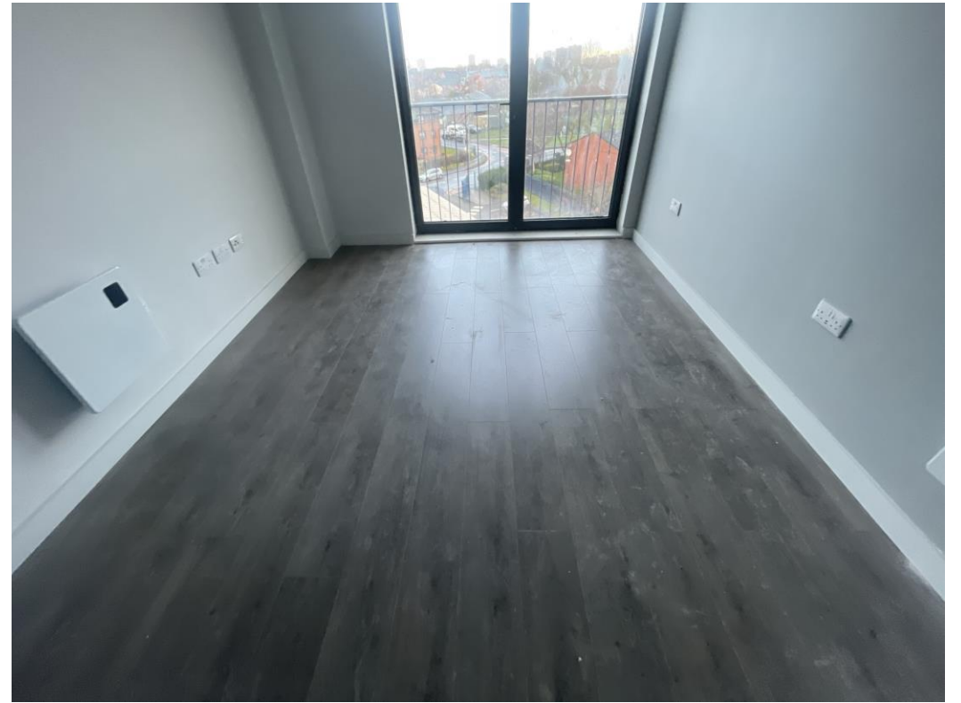
Level 5 – Laminate installed
