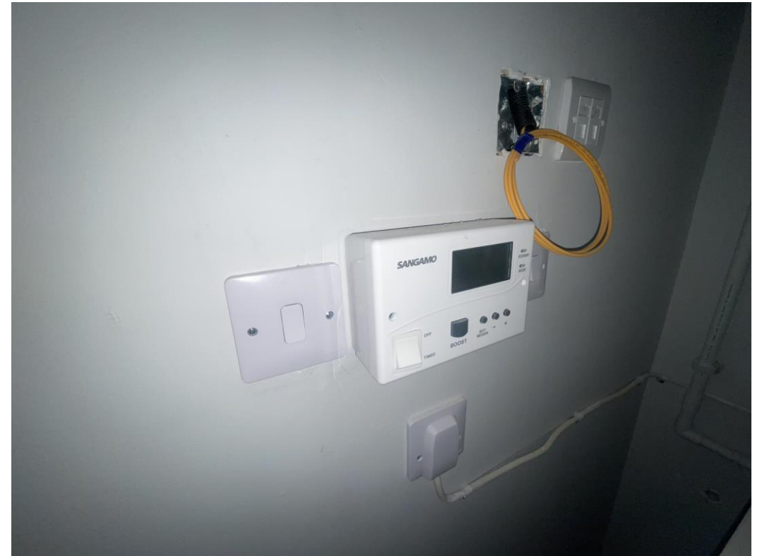
Level 1 – 2 nd fix mechanical controls
