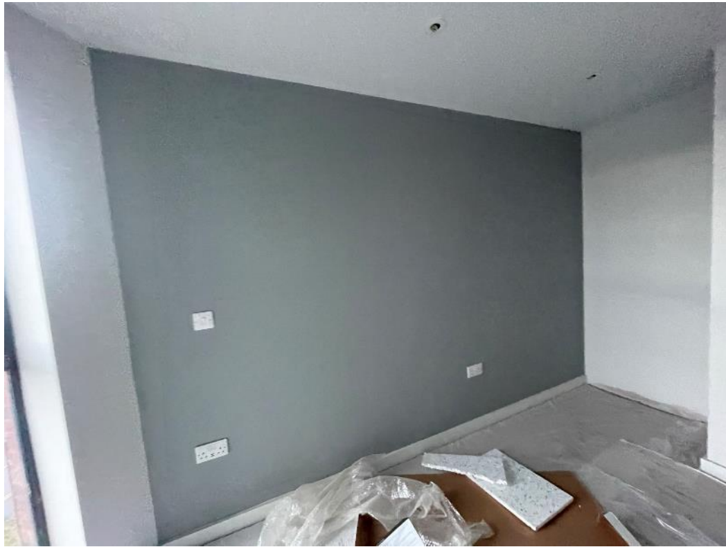
Level 6 – Internal doors installed
