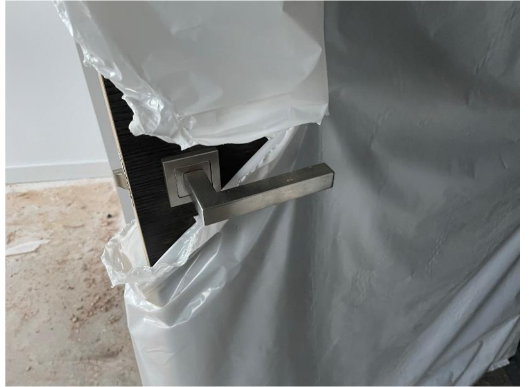
Level 2 – Ironmongery installed
