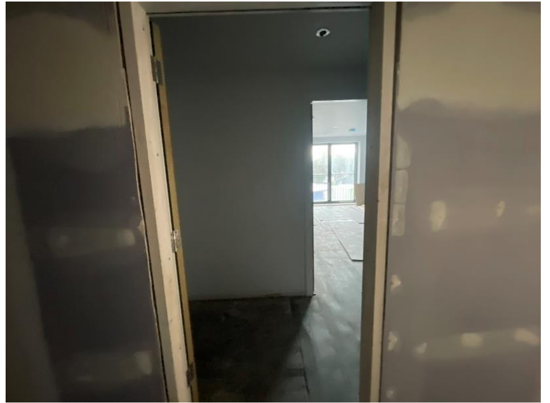
Level 3 – Hoist apartment door frames installed
