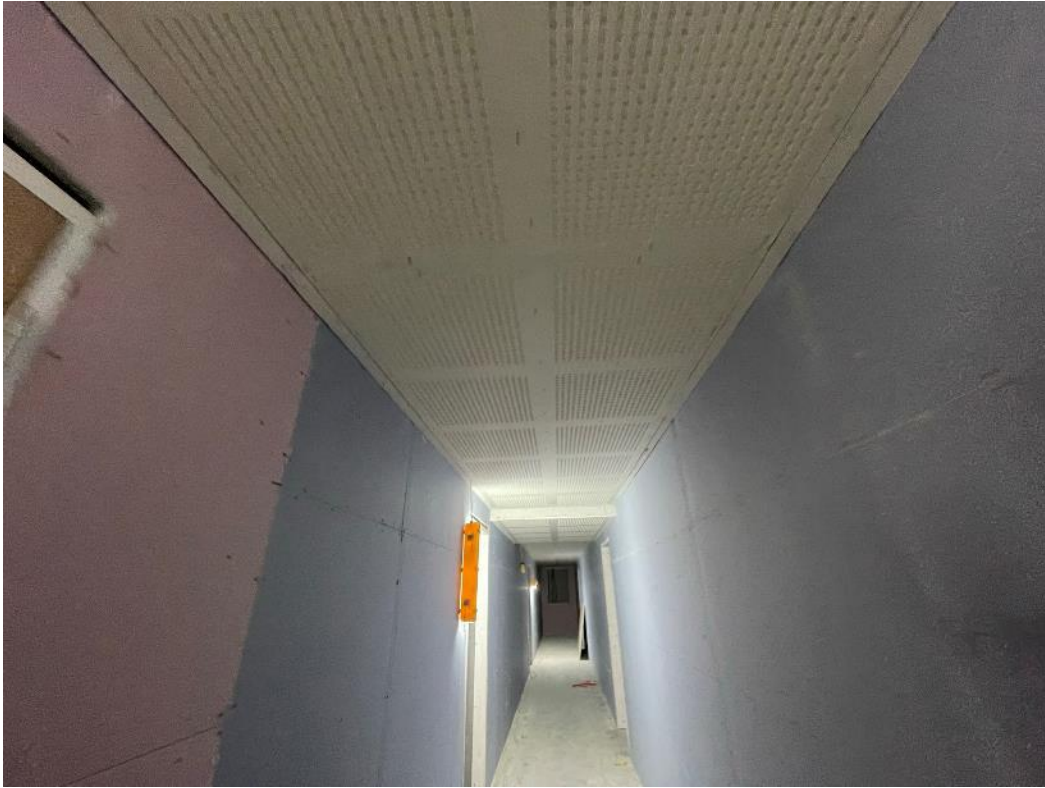
Level 4 – Acoustic ceiling decoration corridor
