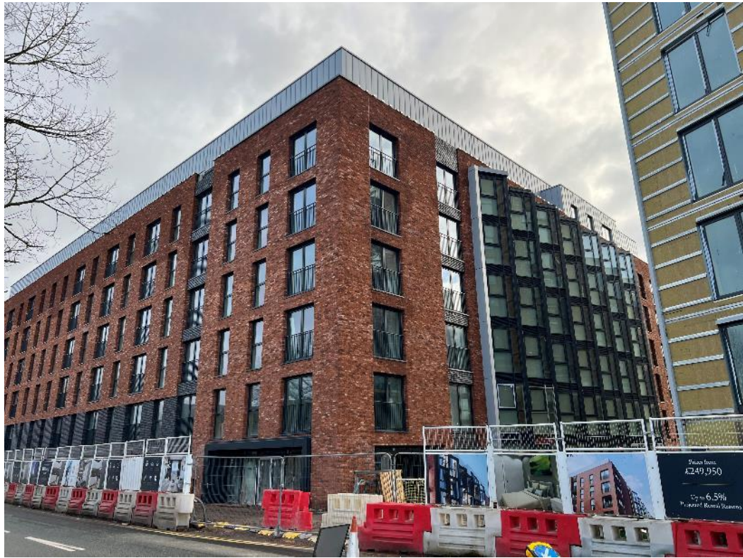
Ordsall Lane site view
