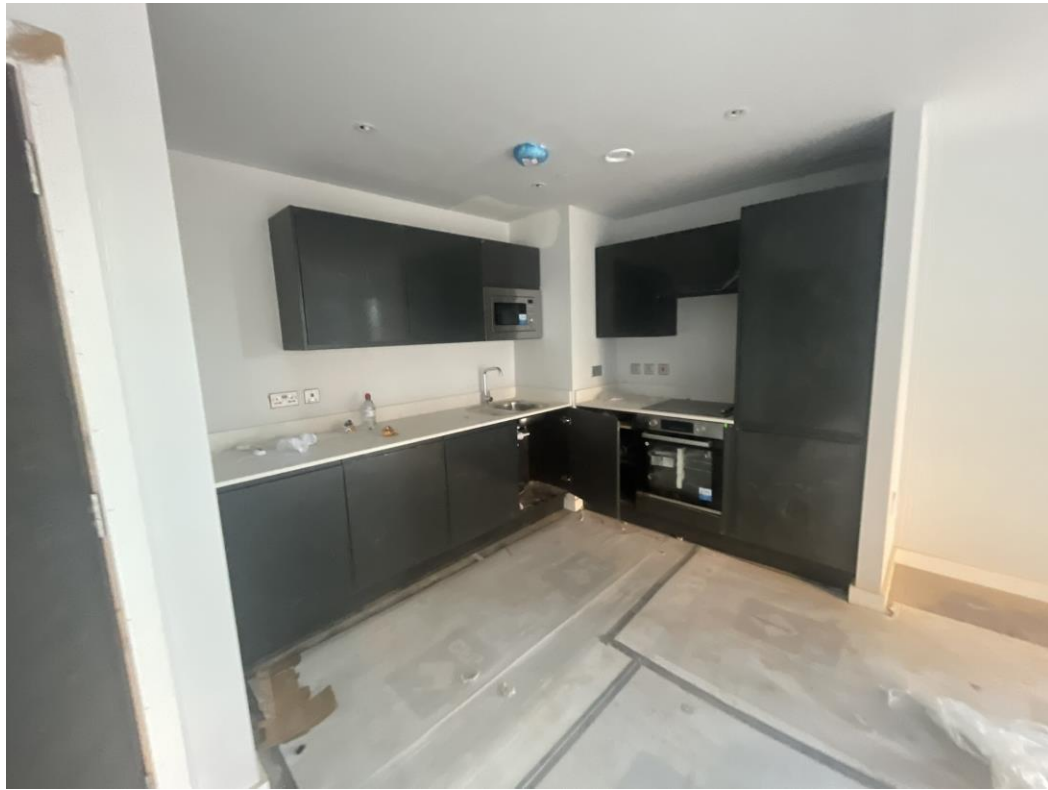
Level 1 – Kitchen units installed
