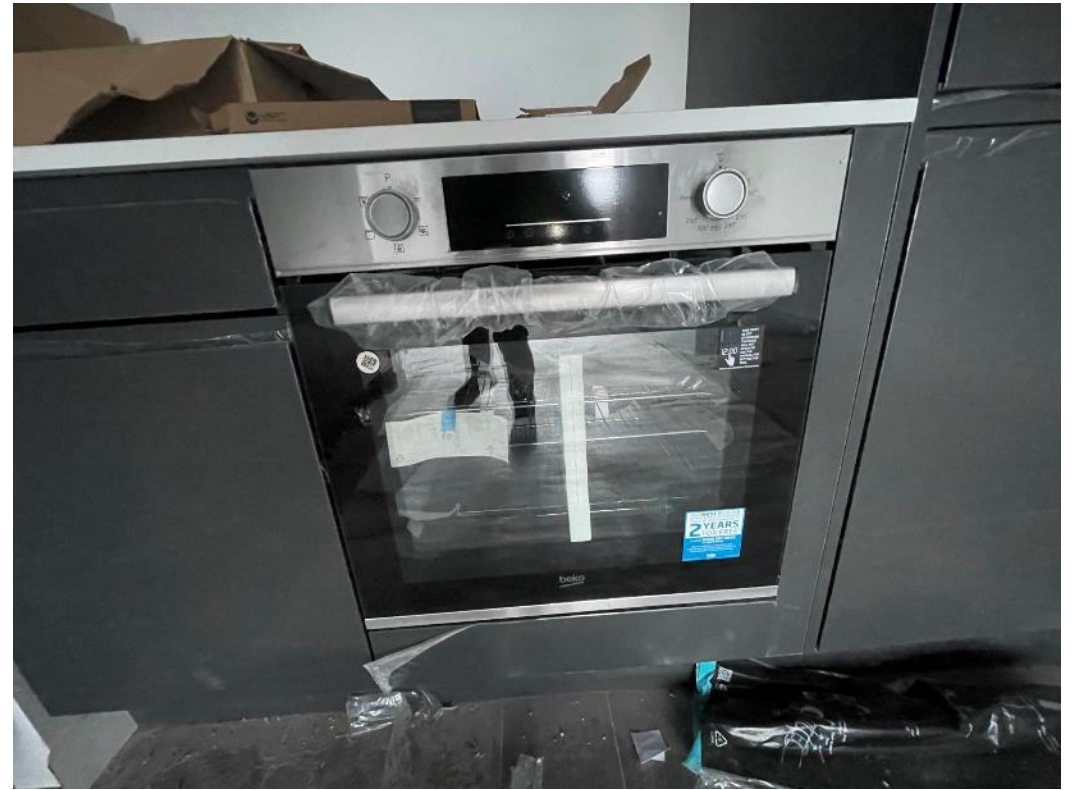
Level 8 – Appliances installed
