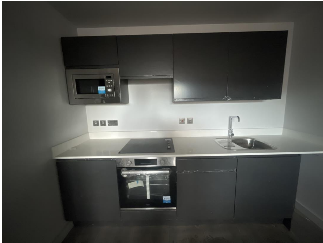
Level 6 – Kitchen units & worktop installed
