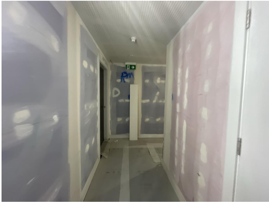
Level 3 – Corridor walls tape & jointed
