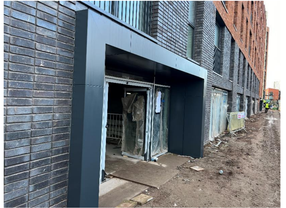
Cladding installed to entrance canopy
