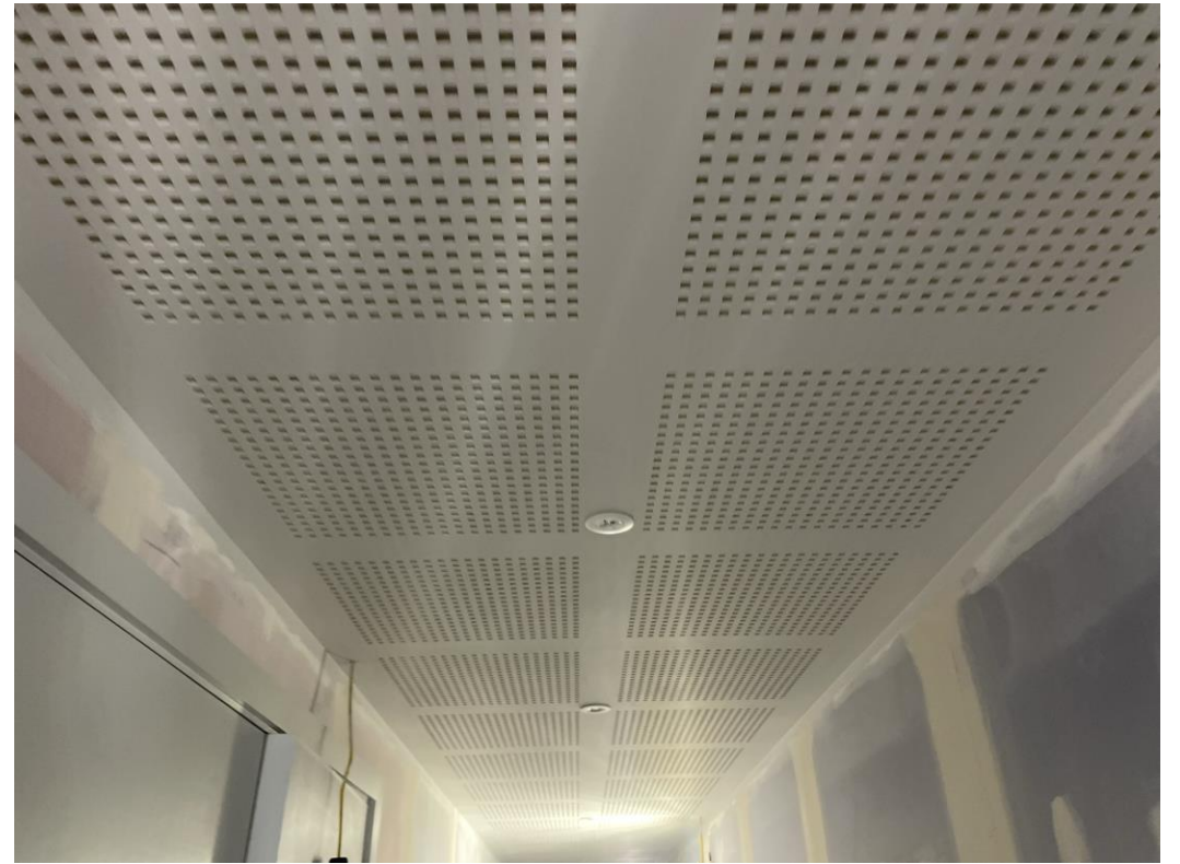
Level 6 – Acoustic ceiling decoration corridor
