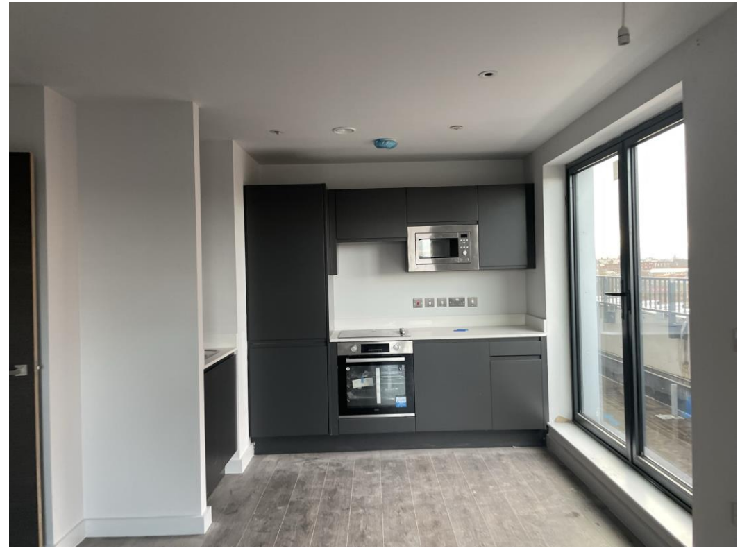
Level 4 – kitchen units & worktop installed
