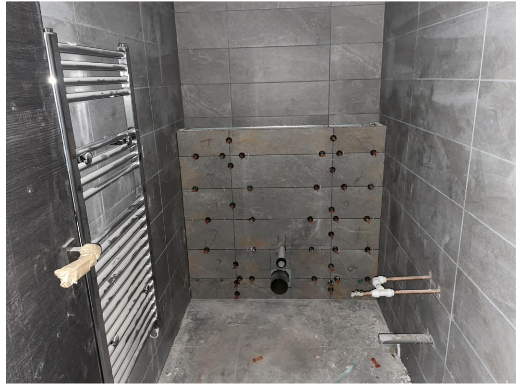
Level 2 – Wall & Floor tiling
