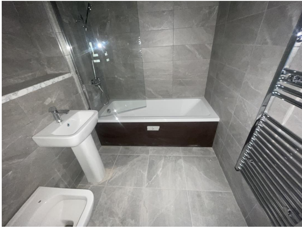
Level 6 – Bathroom shower screen installed
