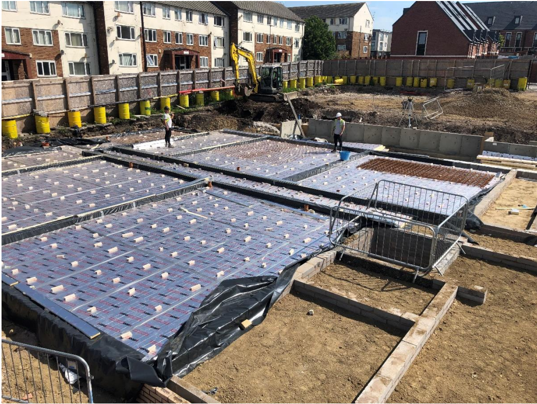
Insulation and sub structure prepared for concrete slab pour
