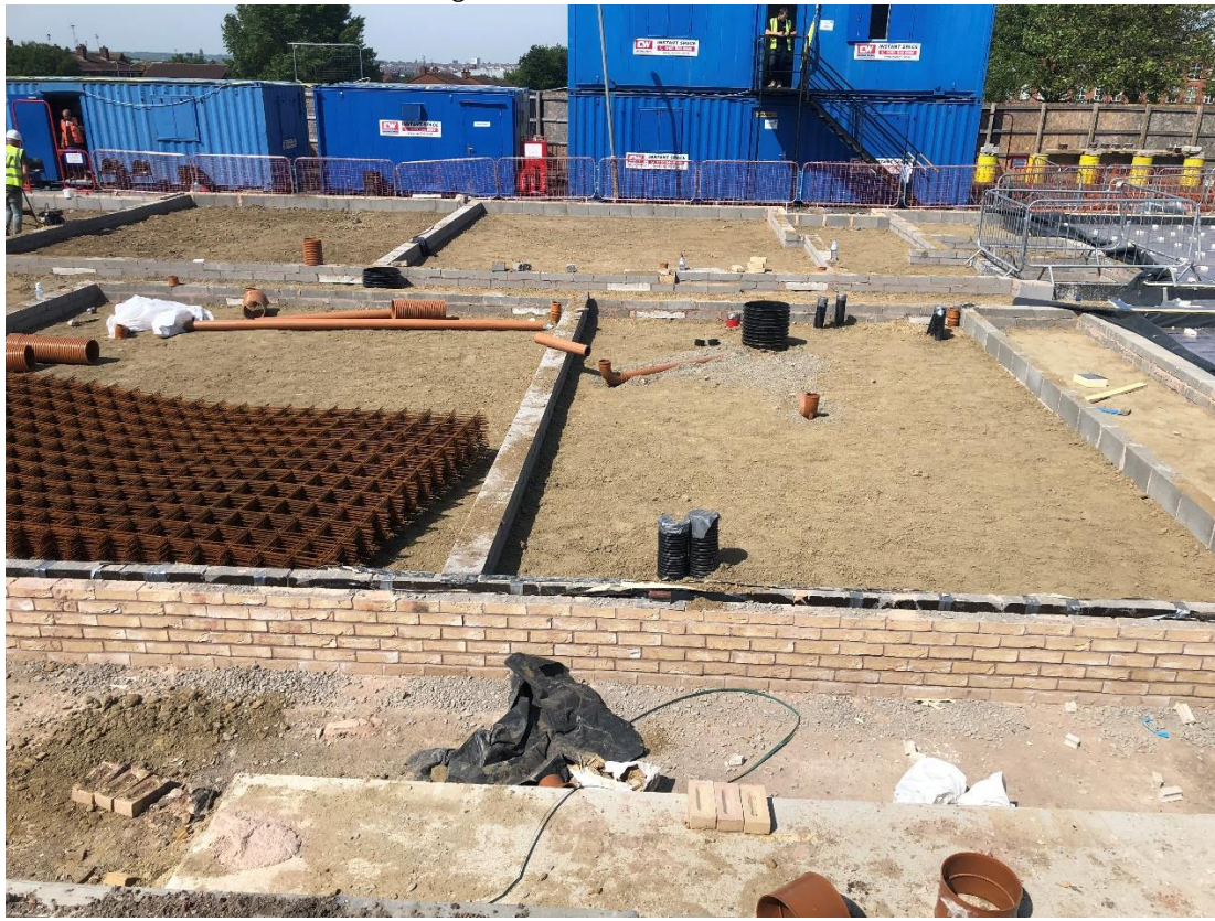
Retaining wall and sub structure brickwork
