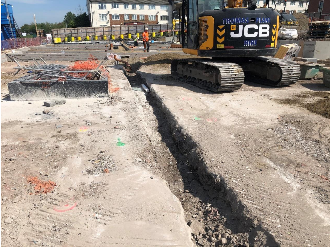
Drainage channels being dug prior to concrete pour
