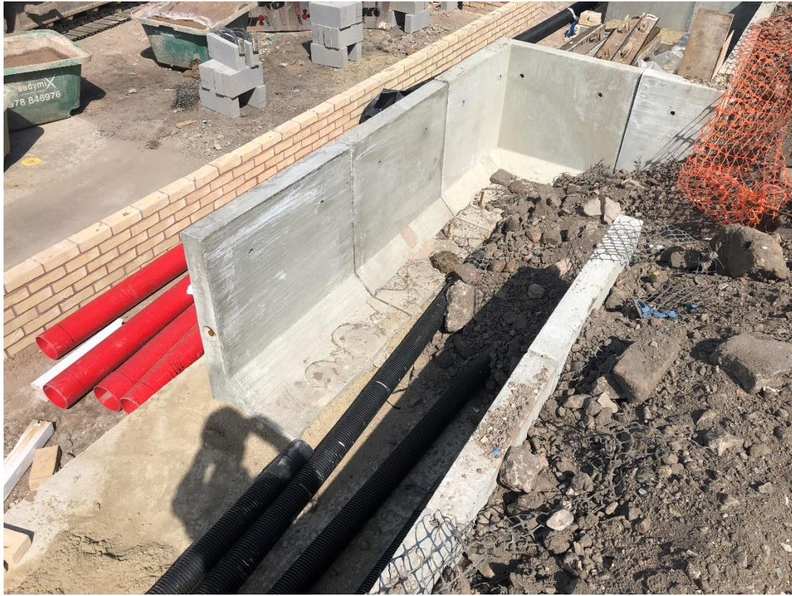
Retaining wall and sub structure brickwork
