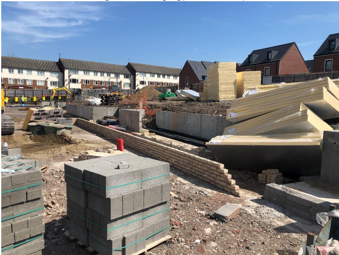
Retaining wall in place and sub structure brick and block
