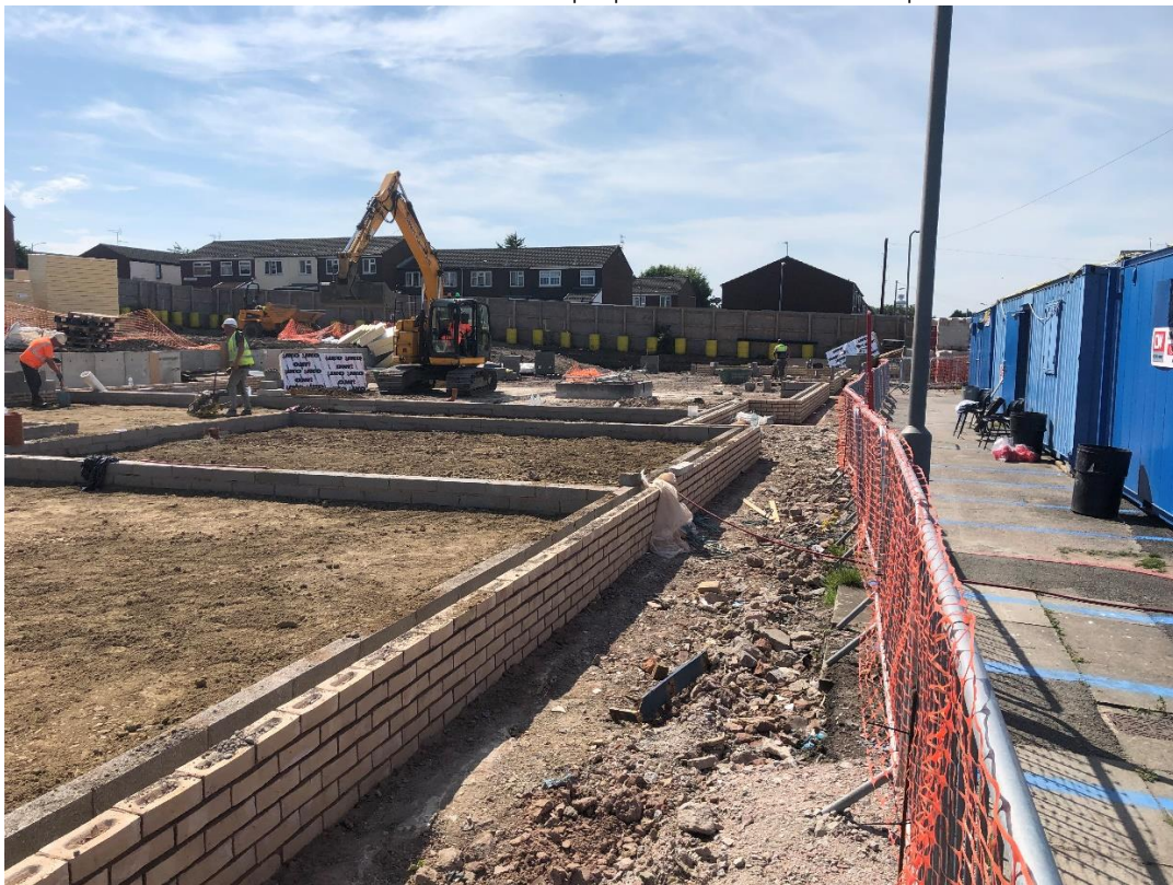
Sub structure brick and blockwork prior to insulation install
