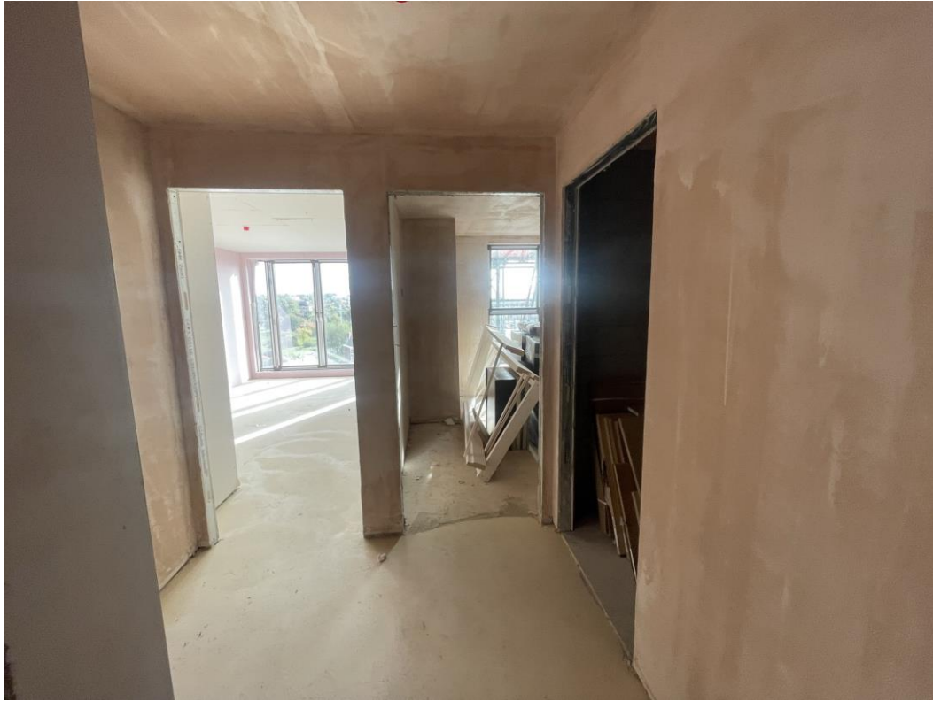
Plaster skim coat ongoing
