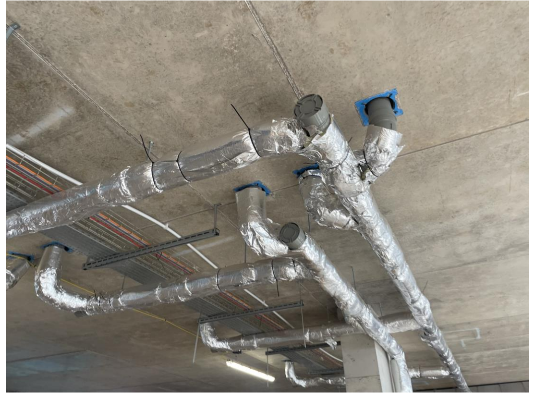
Insulation installed to soil vent pipework
