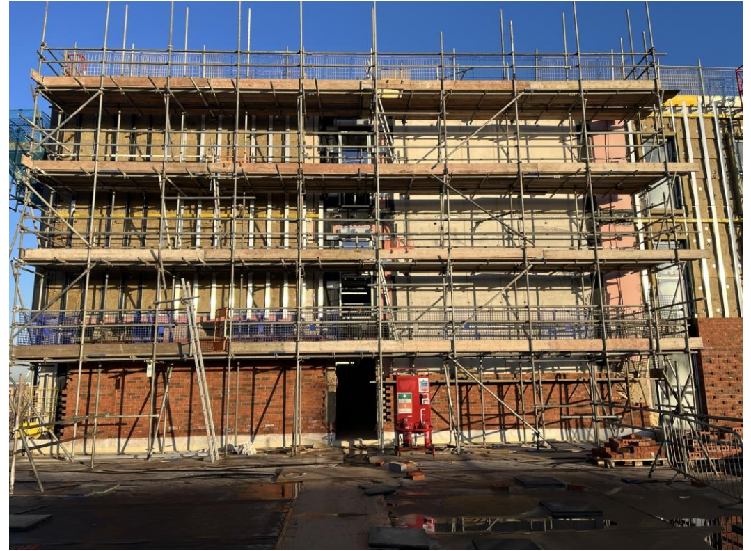
Block D Section A – Viewed from roof terrace
