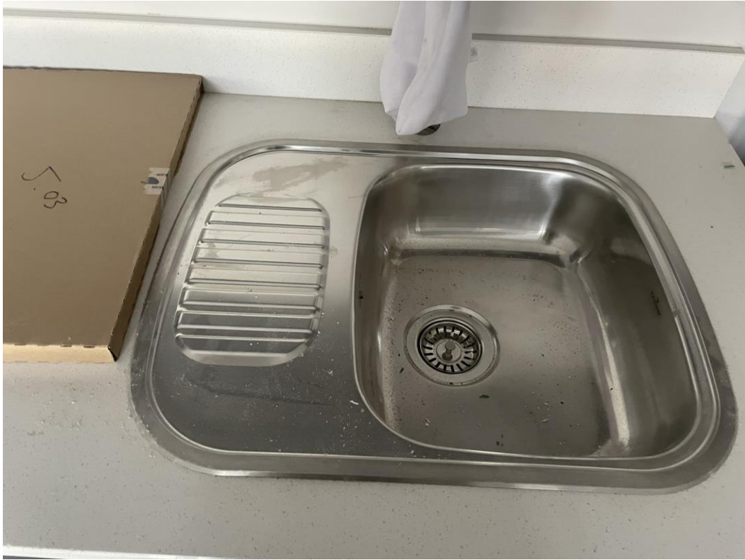
Sink installation ongoing
