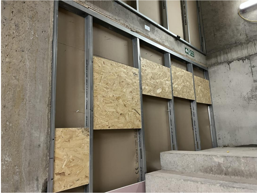
Pattress installation to staircore
