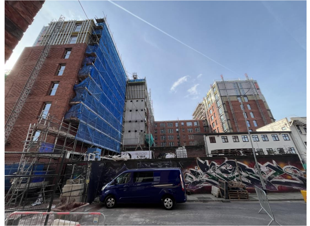
Block D – viewed from Block B podium
