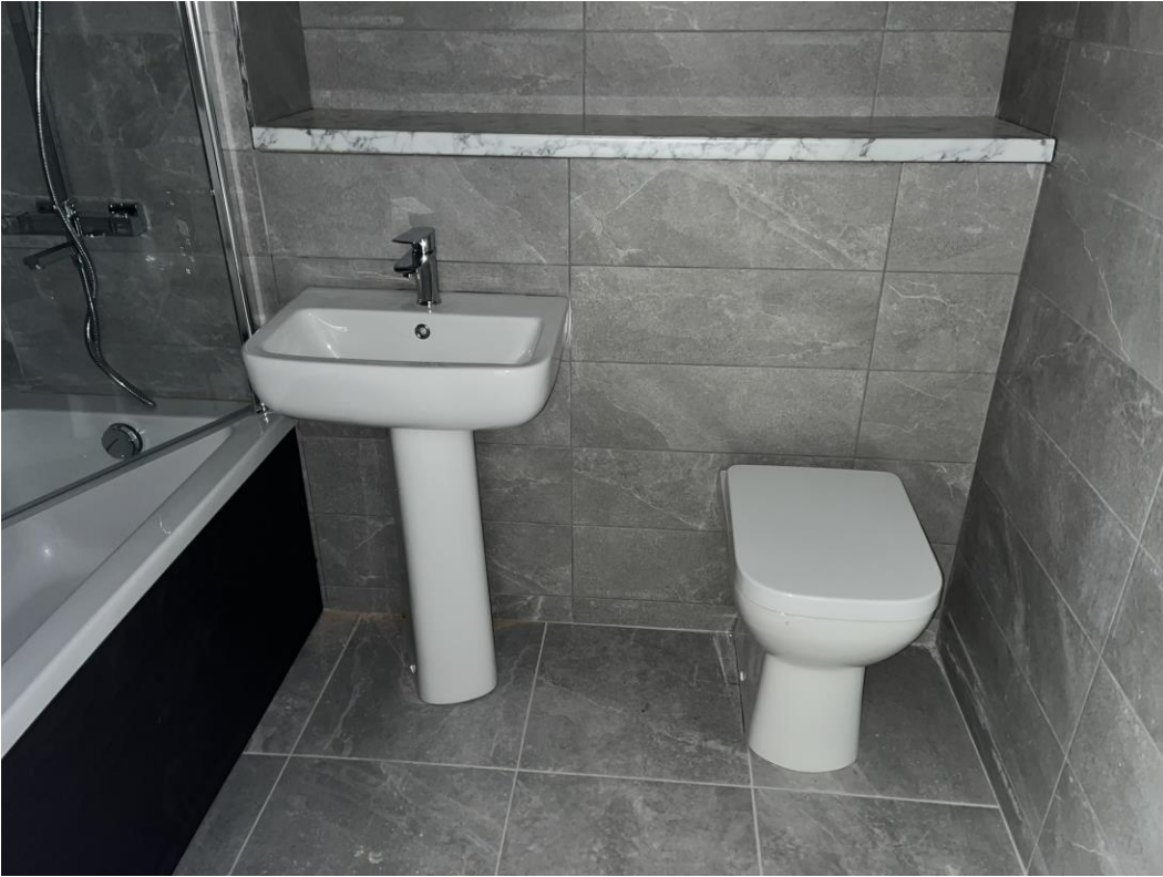
Sanitary installation ongoing
