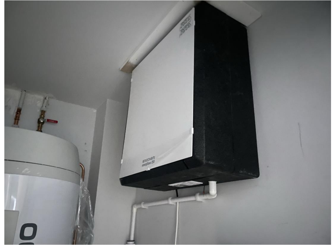
Ventilation installation ongoing
