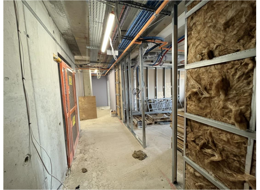
Hoist apartment close-ups ongoing
