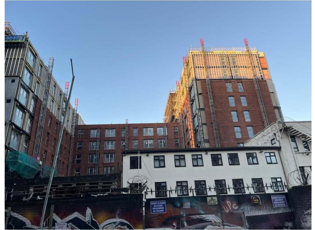
Block D Section A & C – Viewed from Crump Street
