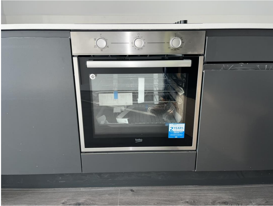
Appliance installation ongoing
