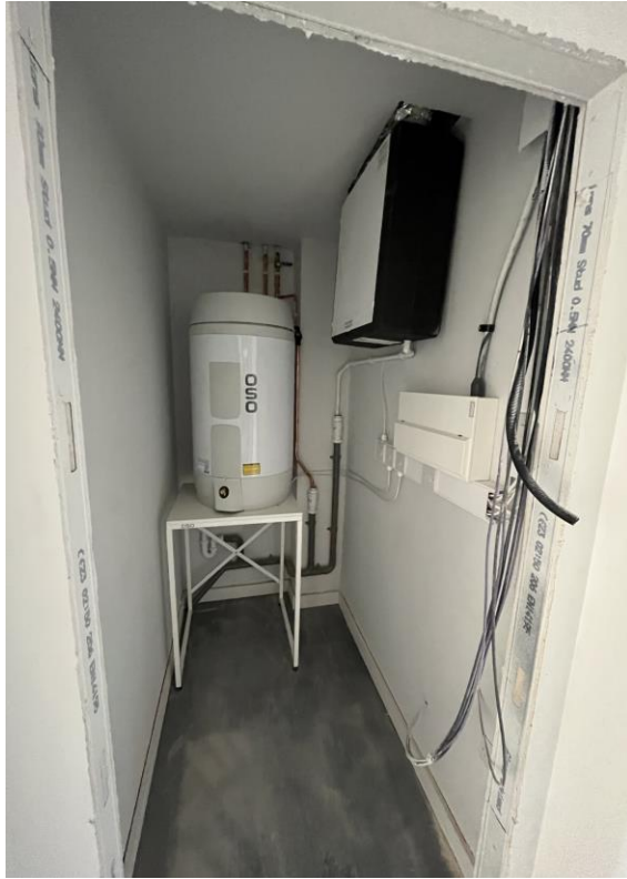
M&E installation progressing
