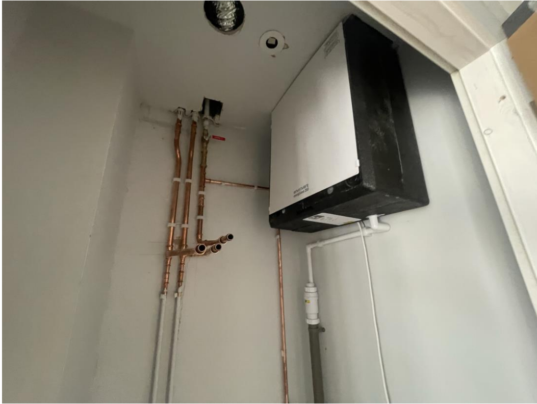
Ventilation installation ongoing
