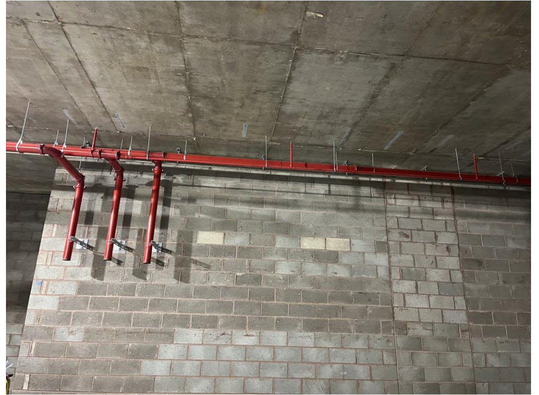
Commercial sprinkler system installation ongoing
