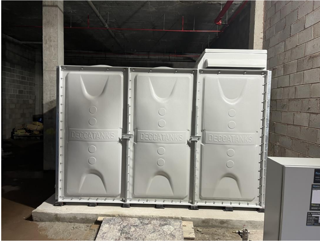
Water tank installation ongoing
