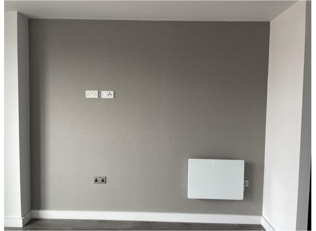
Wall covering installation ongoing
