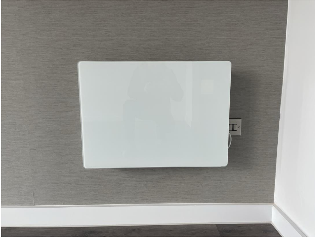
Electrical heater installation ongoing
