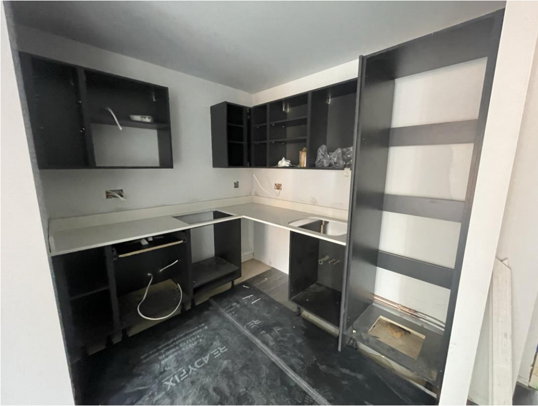
Kitchen installation ongoing
