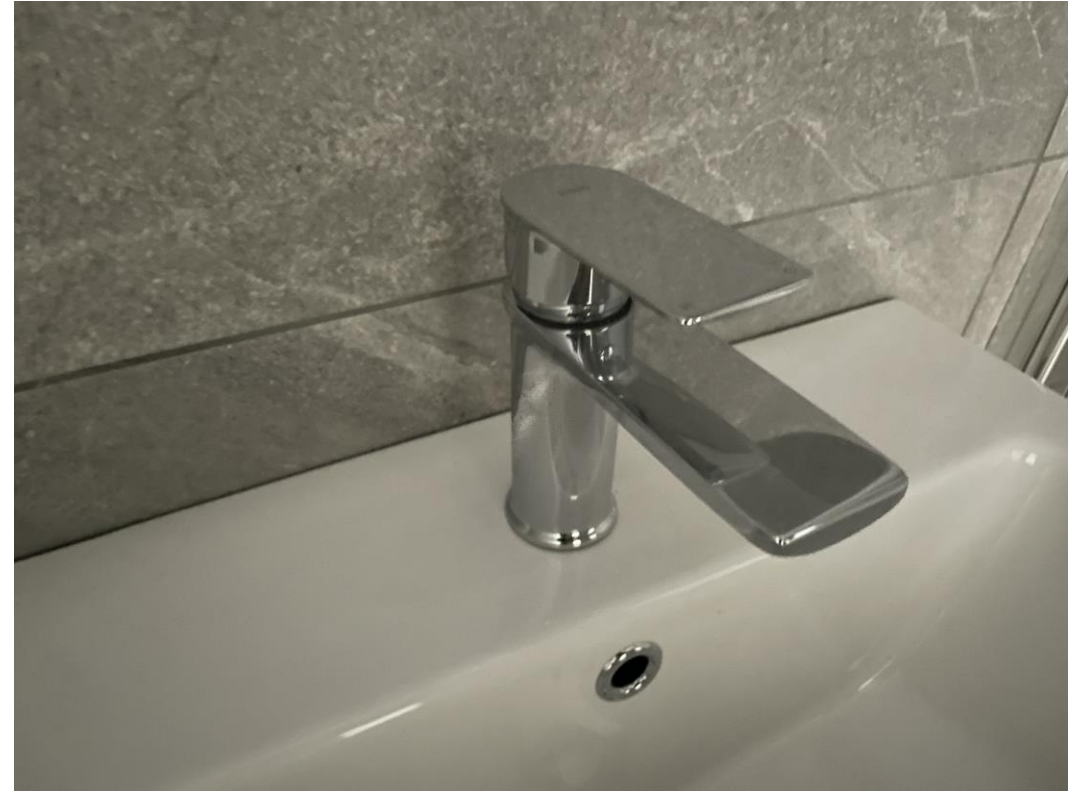
Sanitary installation ongoing
