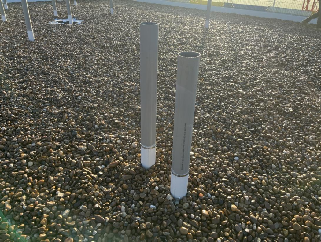
Block D Section A – Soil vent pipe installation
