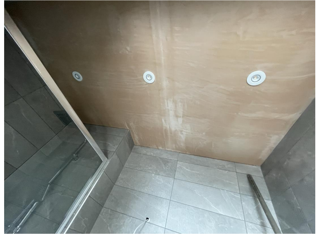
Plaster skim coat ongoing
