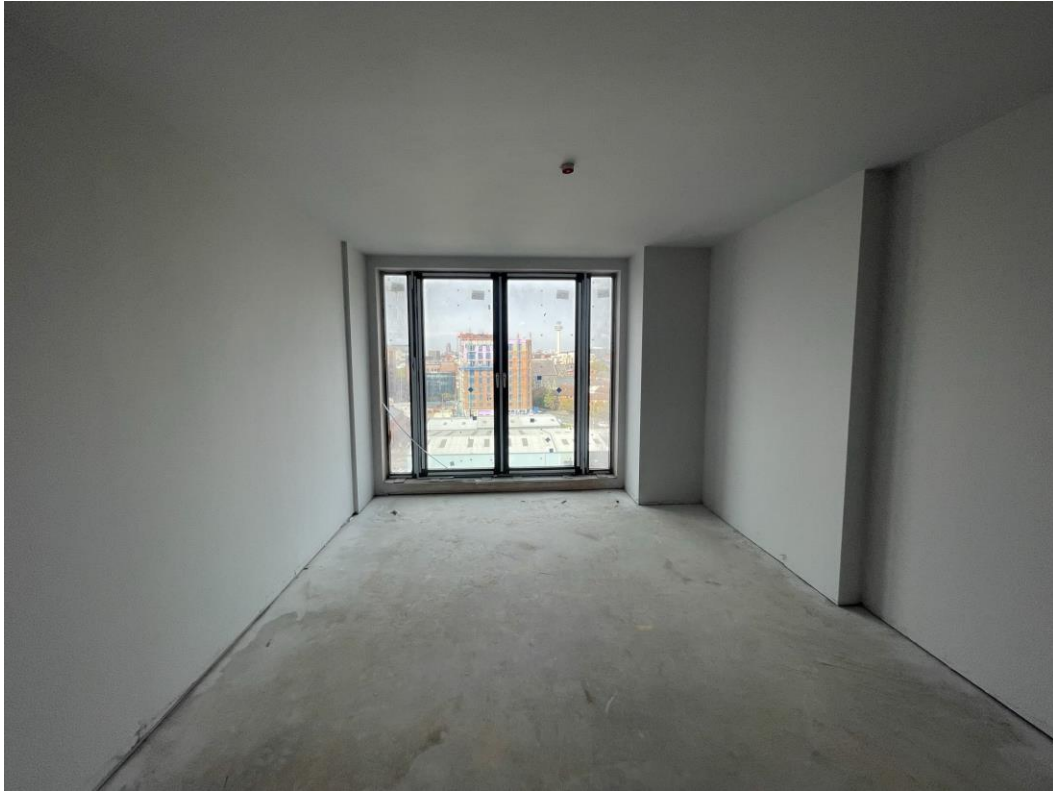
Mist coat application ongoing
