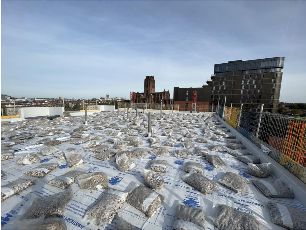
Block D Section A – Roof installation progressing
