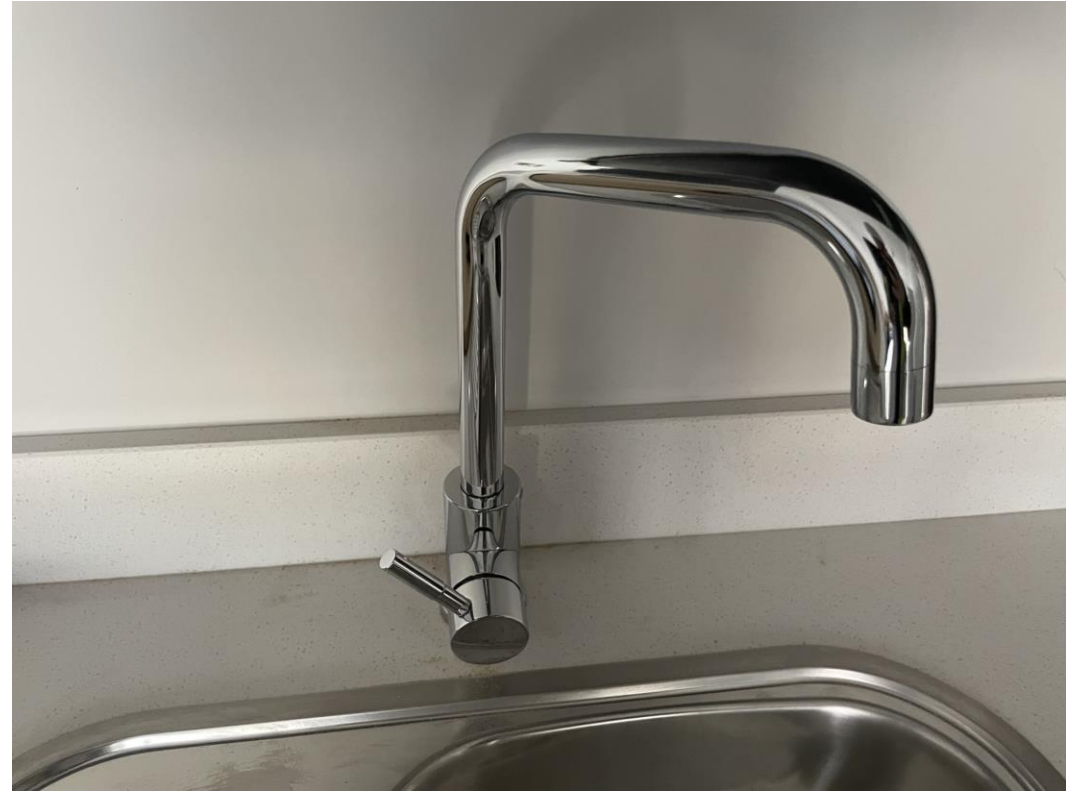
Tap installation ongoing
