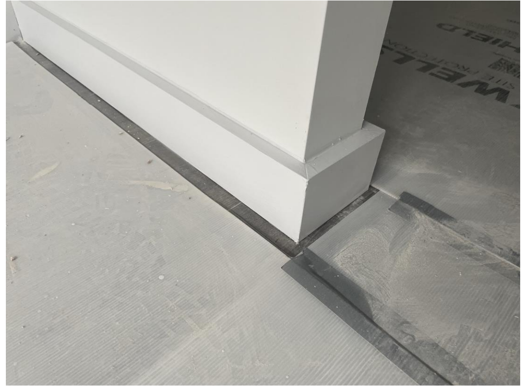
Skirting board installation ongoing
