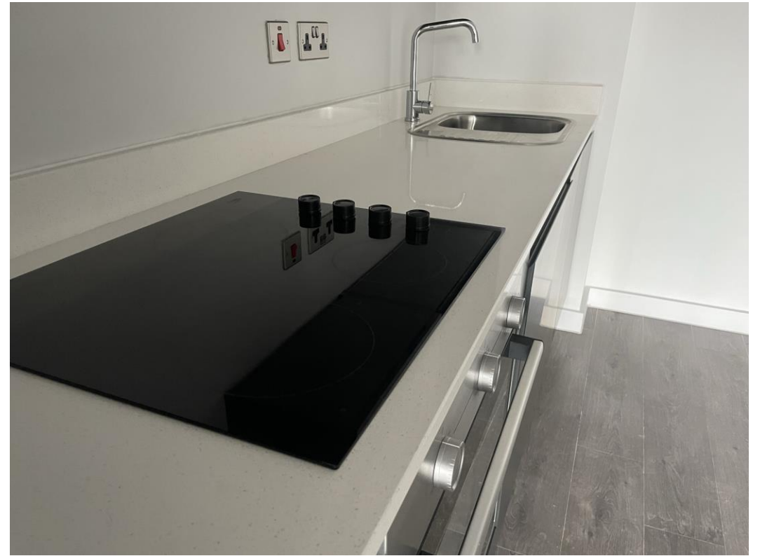
Appliance installation ongoing
