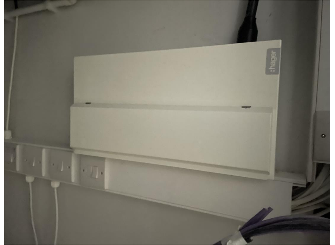
Distribution installation ongoing
