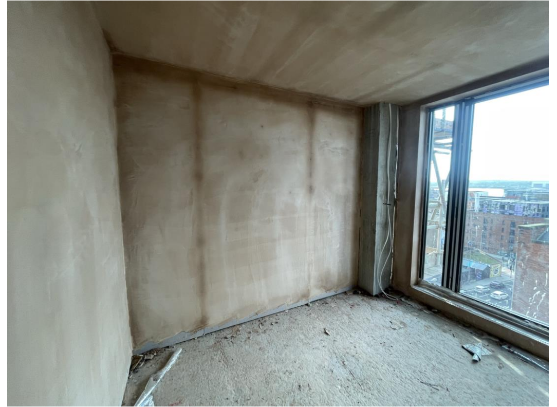
Plaster skim coat ongoing
