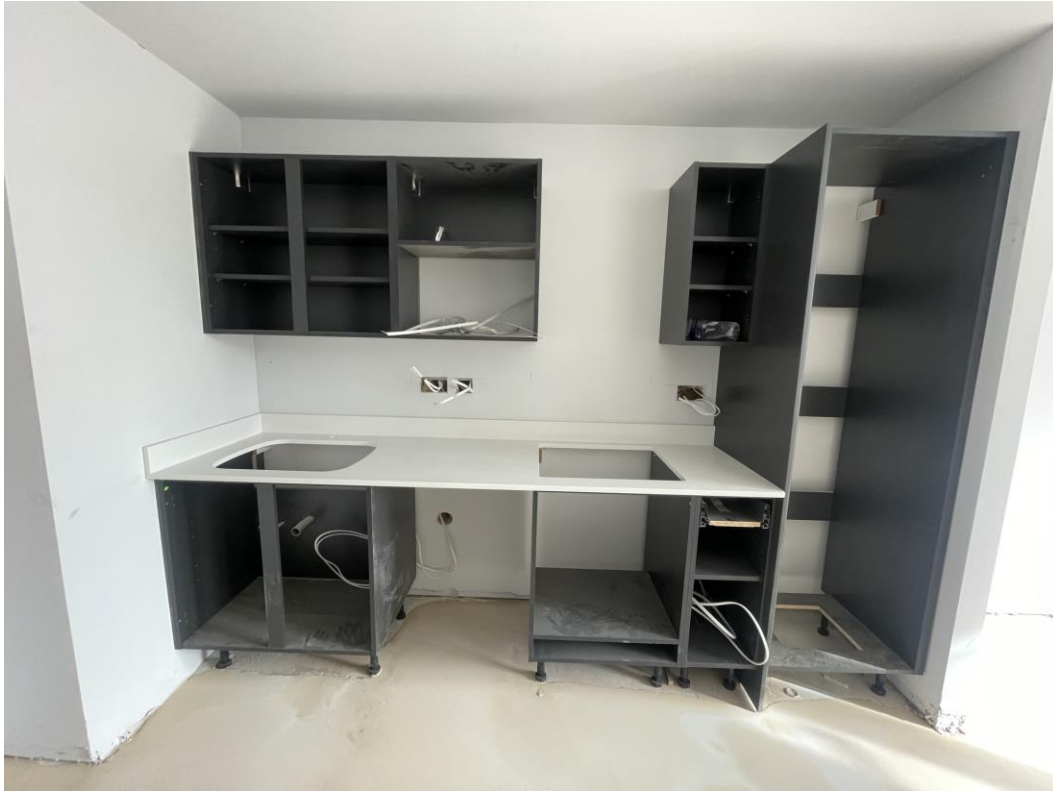
Installation of kitchen units ongoing
