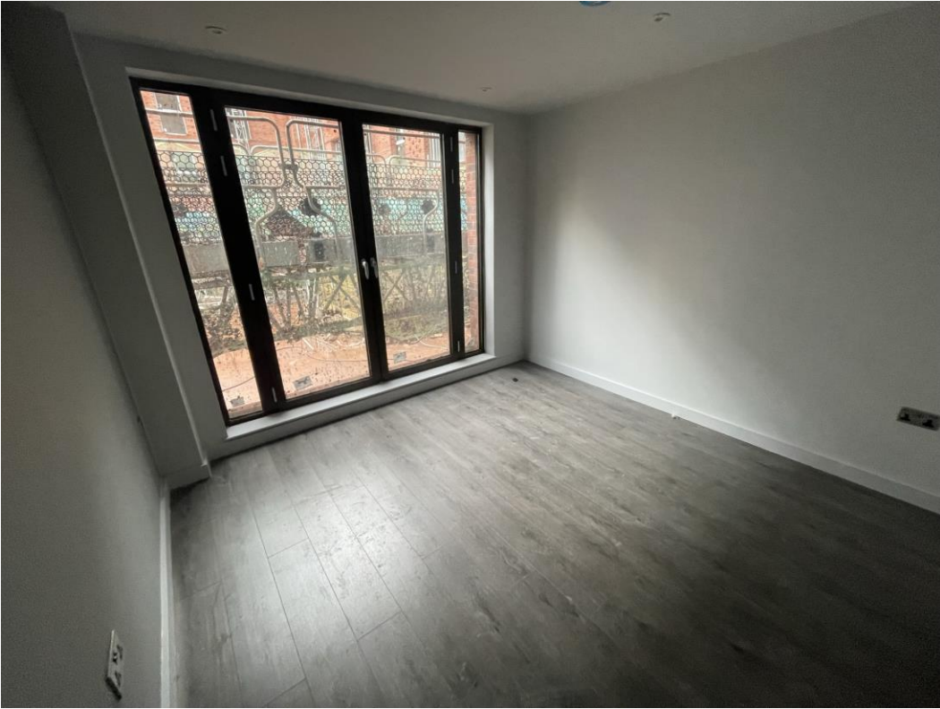
Laminate flooring installation ongoing
