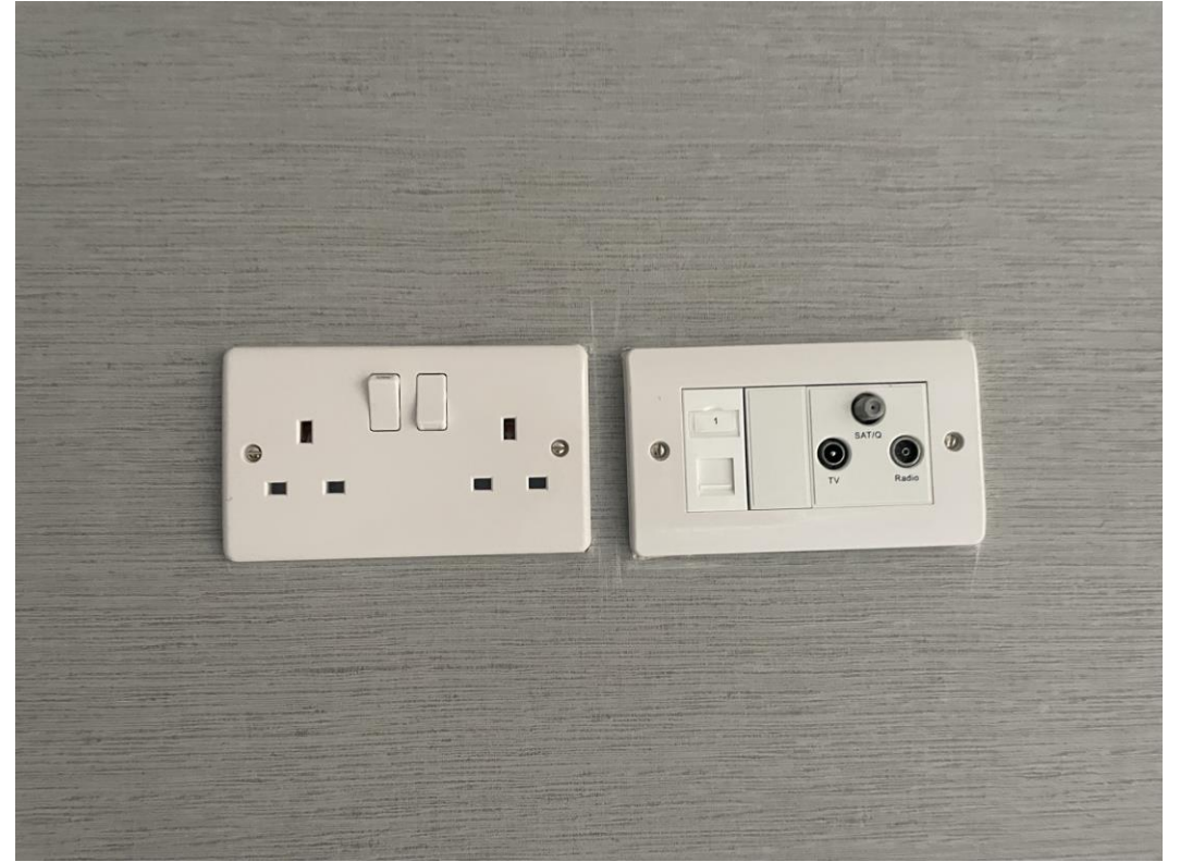
Final fix installation ongoing
