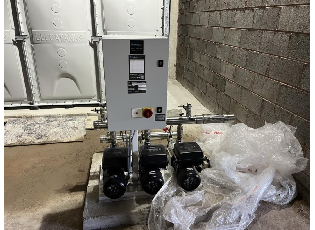
Water tank installation ongoing
