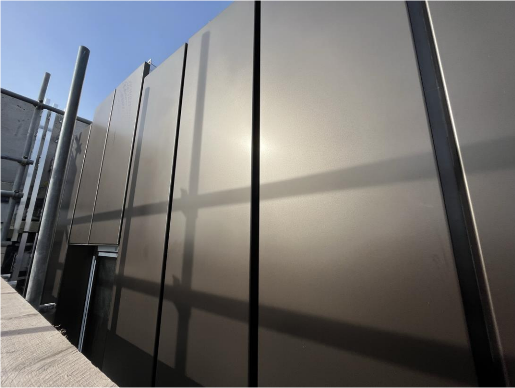
Balcony cladding installation progressed
