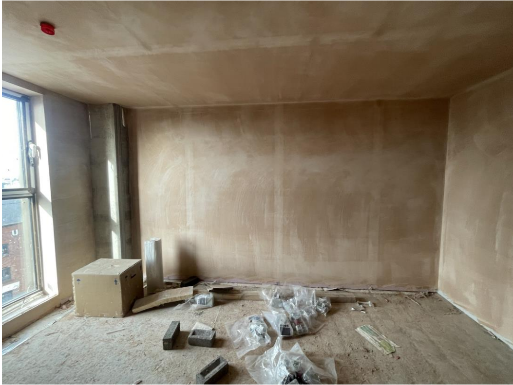
Plaster skim coat ongoing
