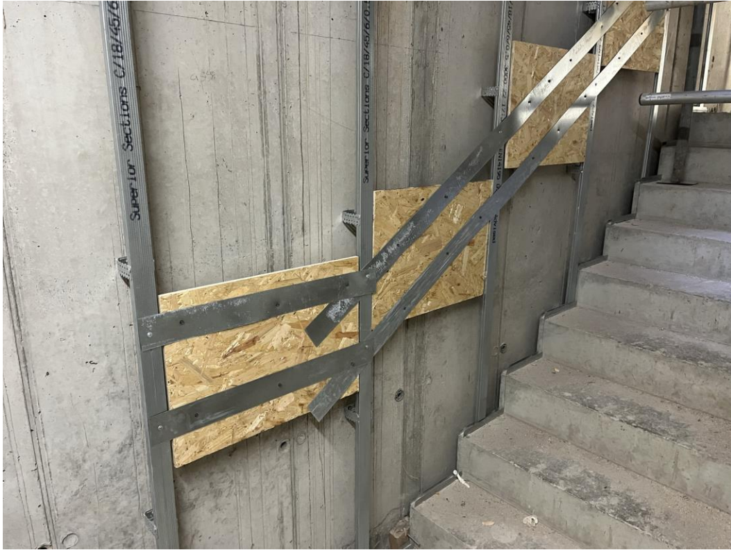
Patress installation to staircore
