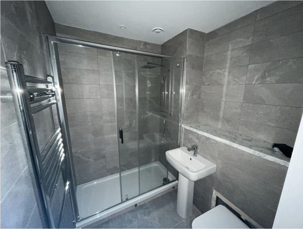
Sanitary installation ongoing
