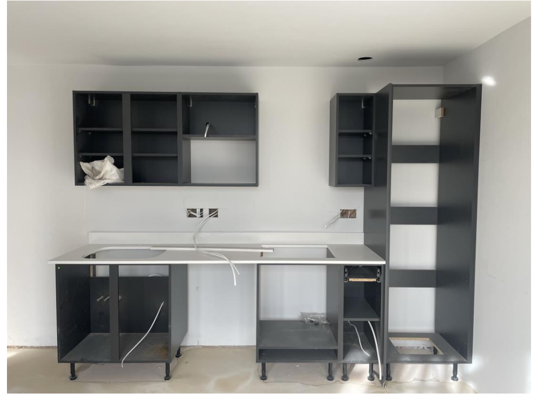
Kitchen installation ongoing
