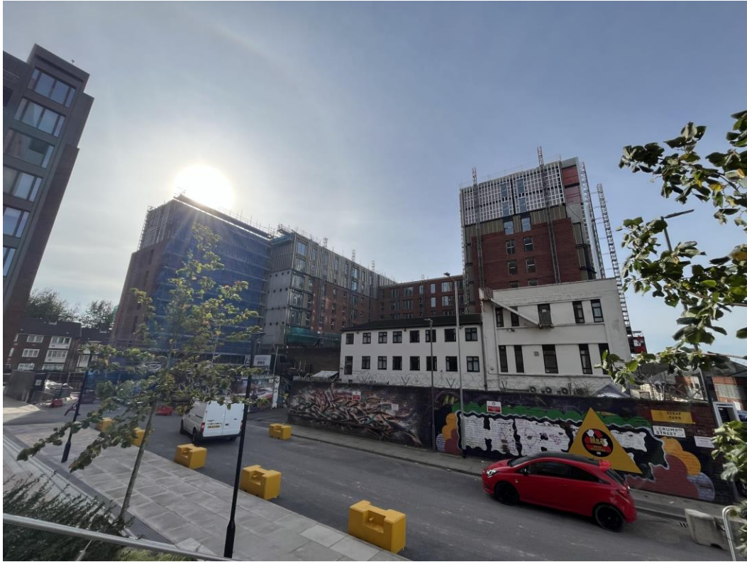
Block D – viewed from Block B podium
