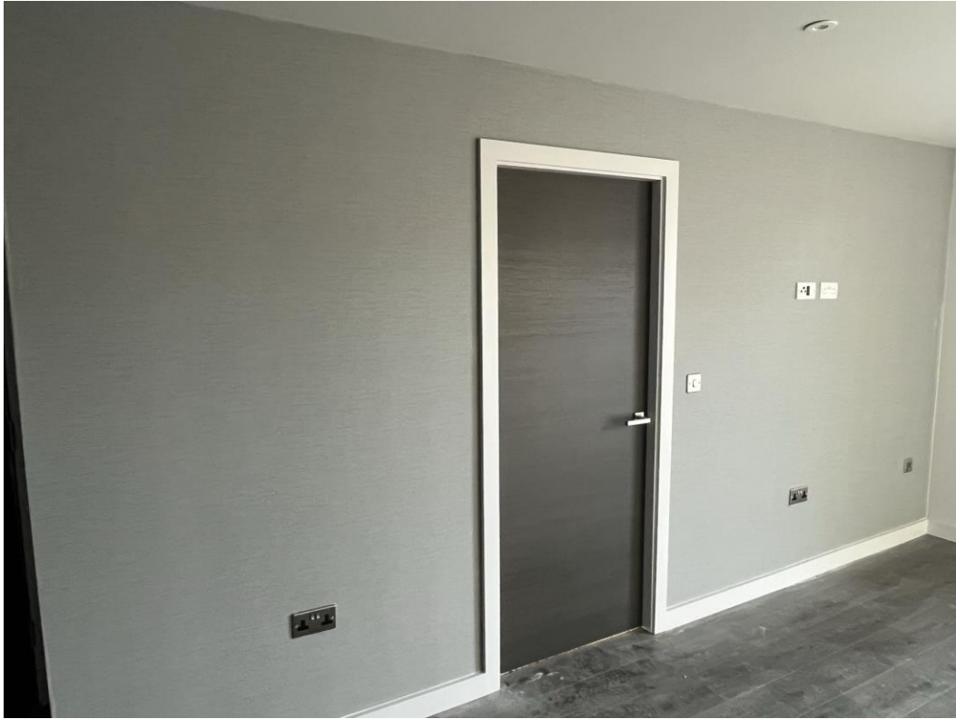
Wall covering installation ongoing
