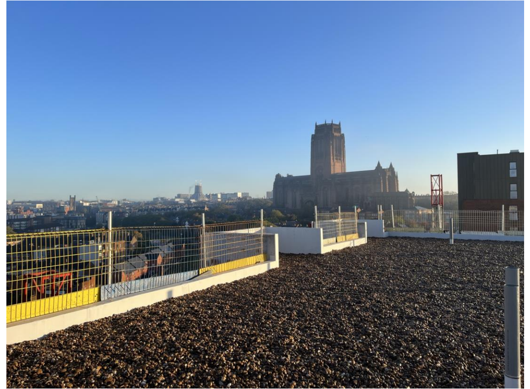
Block D Section A – Roof installation complete
