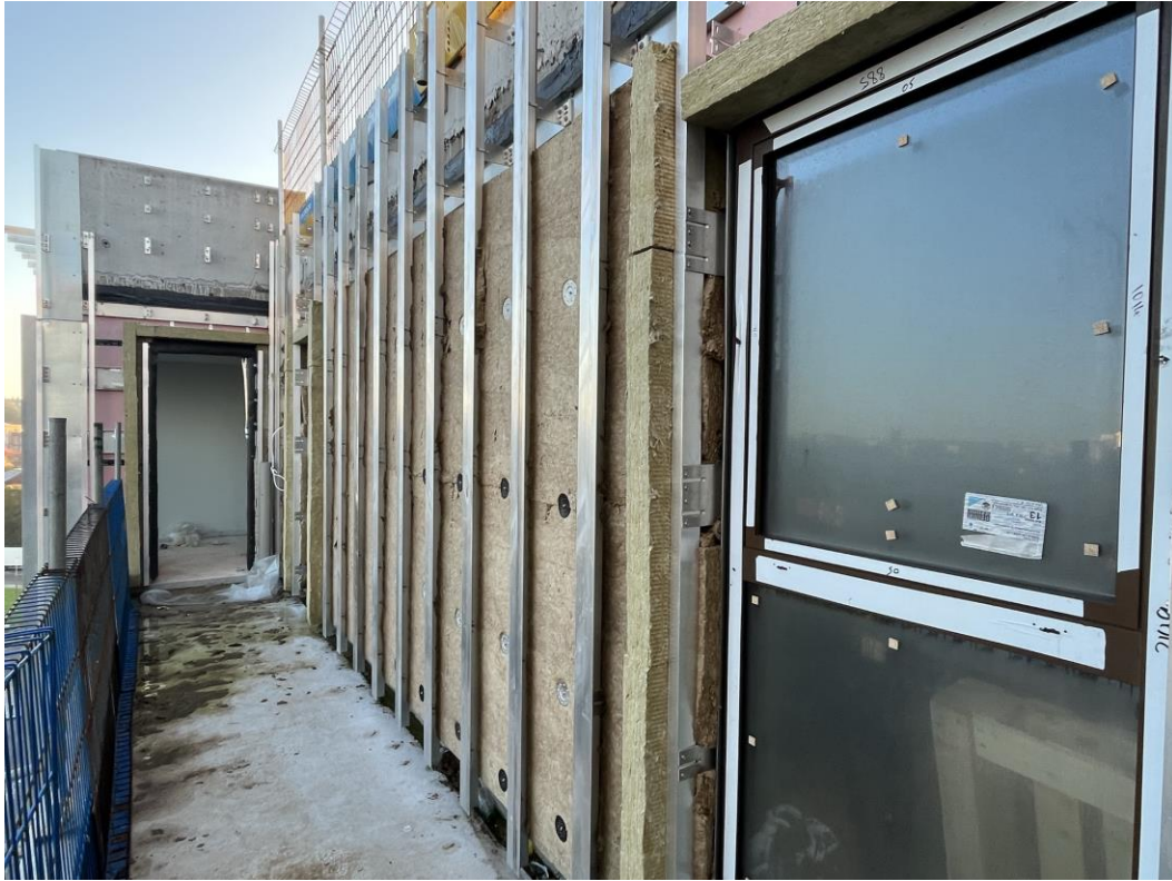
Balcony cladding installation progressed
