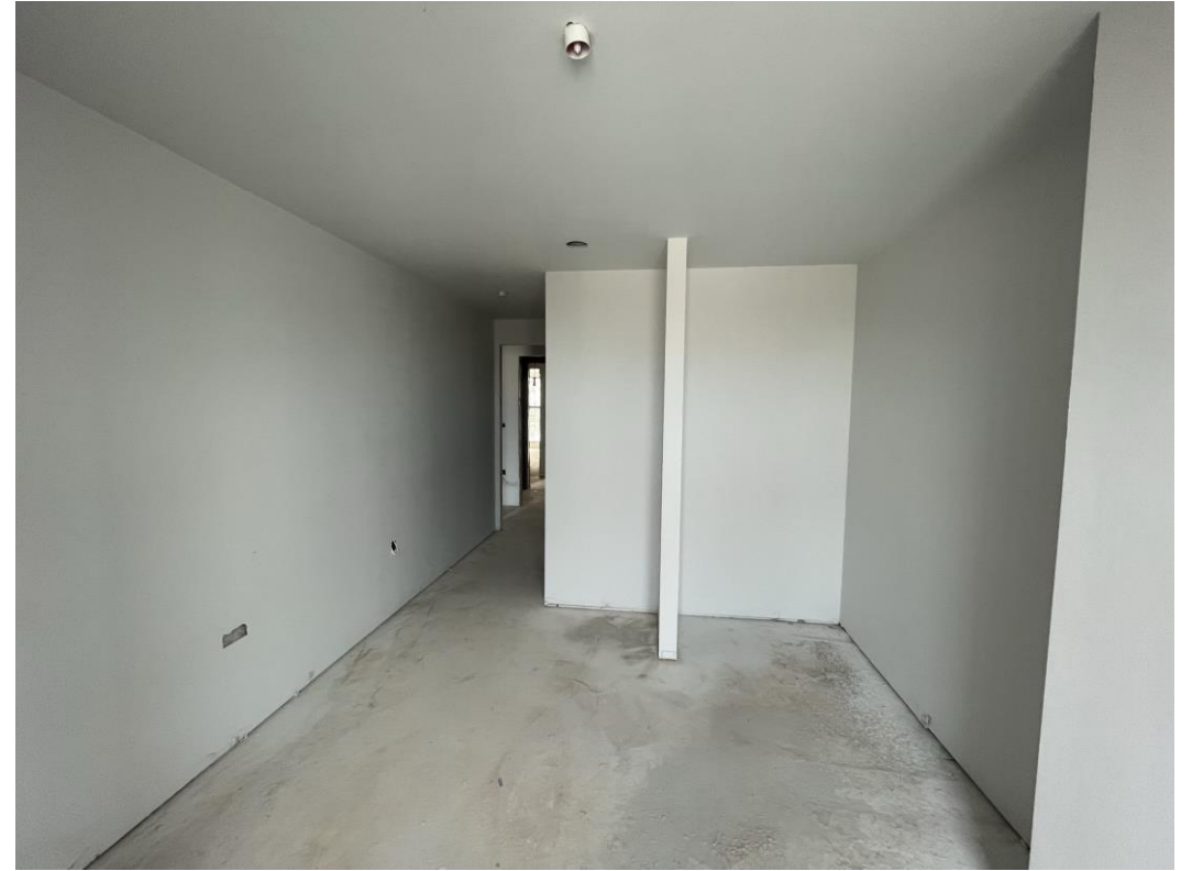
Mist coat application ongoing
