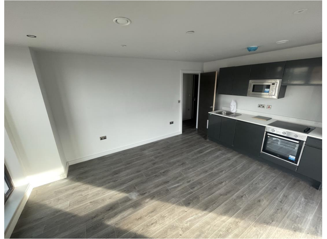
Laminate flooring installation ongoing
