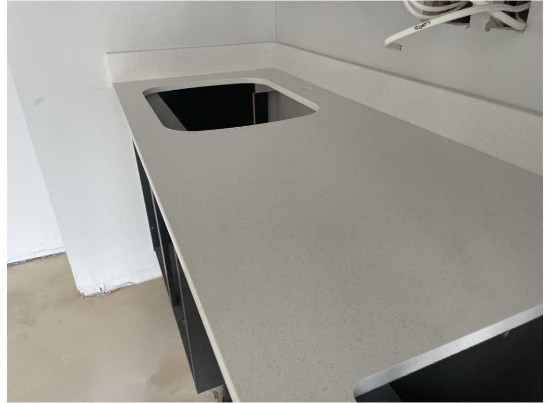
Installation of kitchen worktop ongoing
