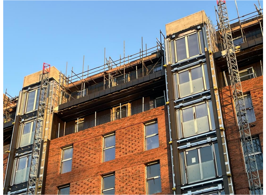
Balcony cladding installation progressed
