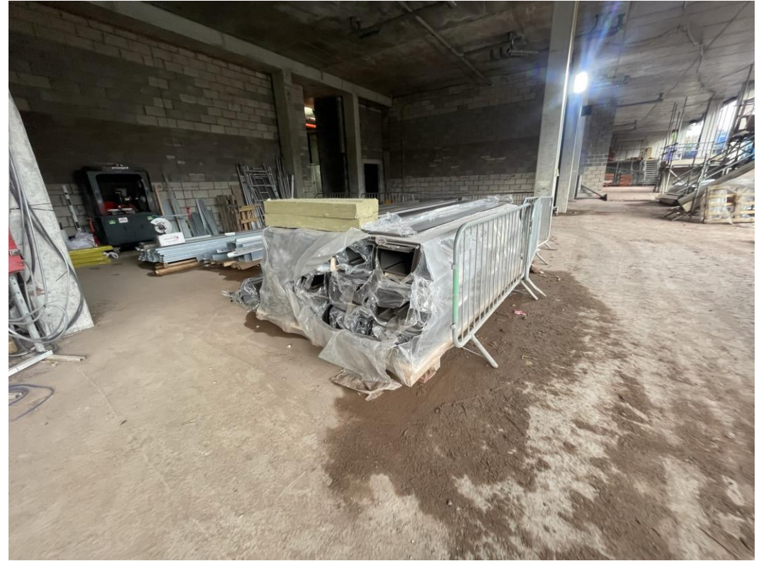
Cladding panels onsite
