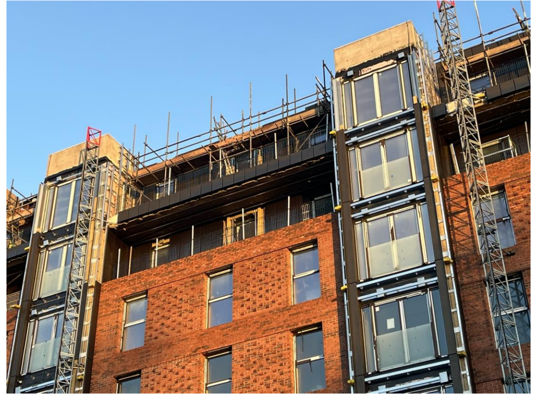
Balcony cladding installation progressed
