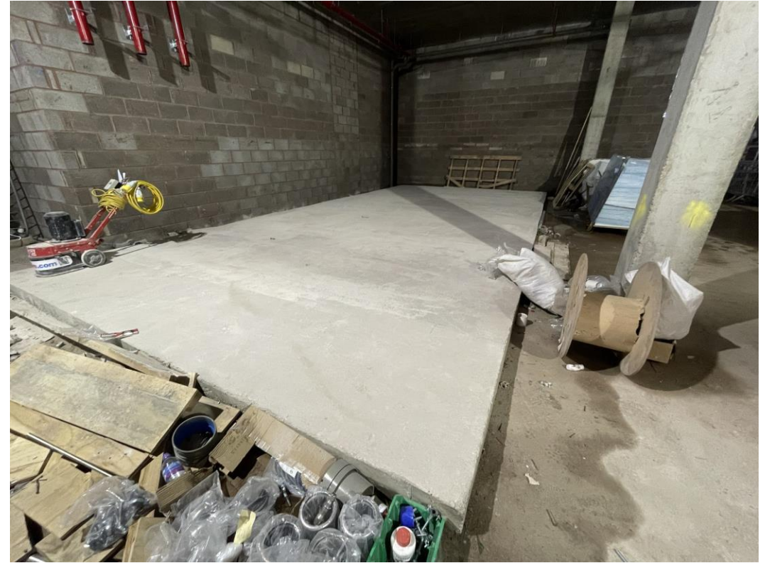
Base for sprinkler tank poured
