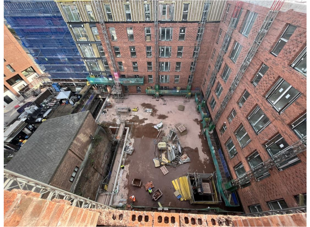
Block D Section C – Podium construction ongoing
