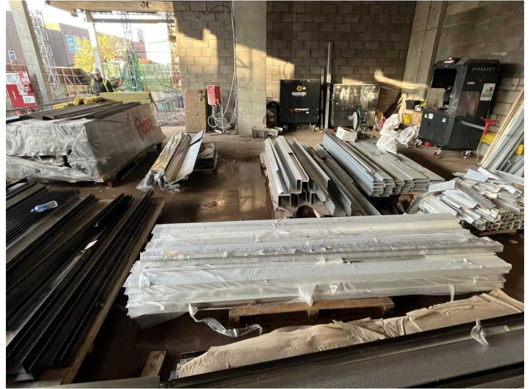
Cladding panels onsite
