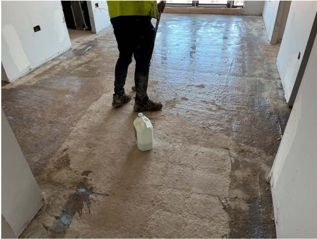
Preparation for screed application ongoing
