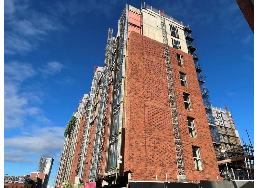
Block D Section B – Brickwork complete to gable end
