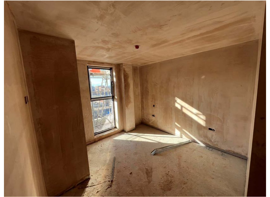
Plaster skim walls and ceiling application ongoing
