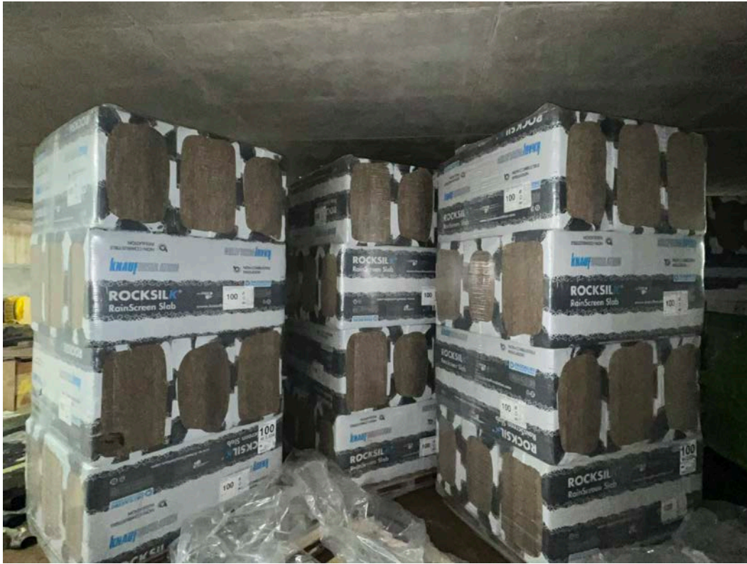
External wall insulation on site
