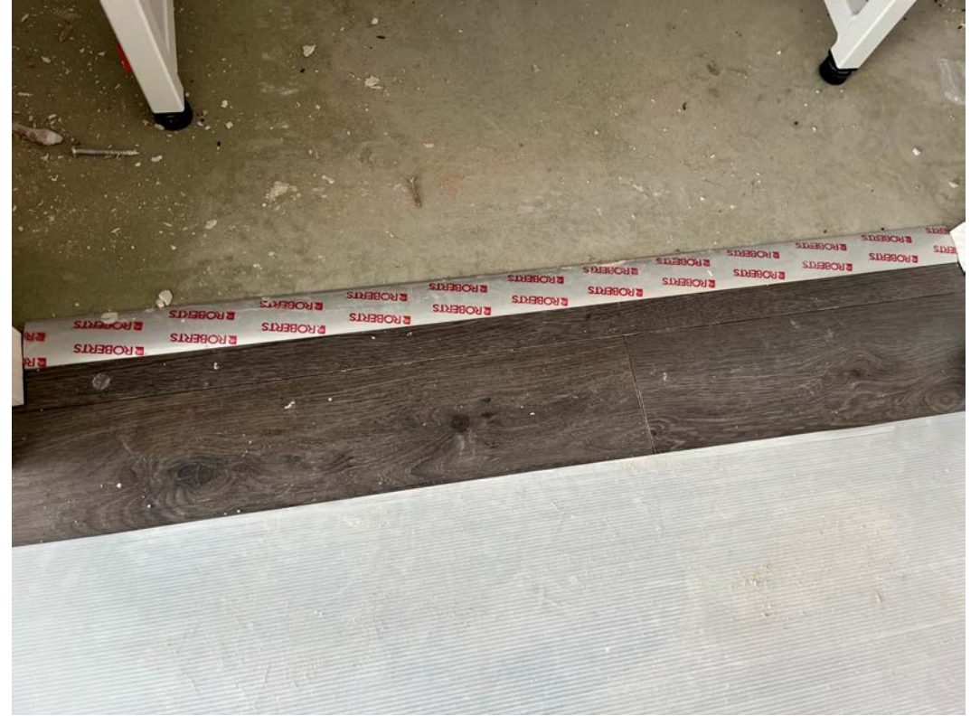
Door threshold strip installation ongoing
