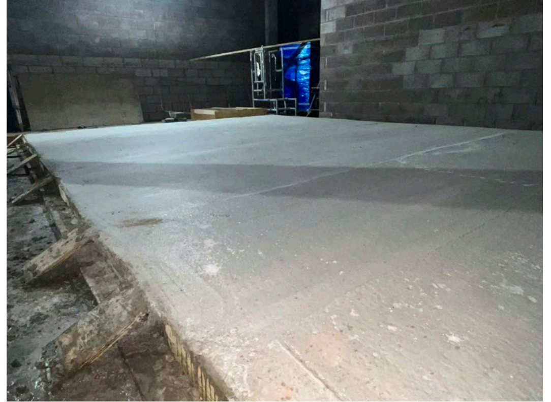
Block D Section A – Concrete slab
