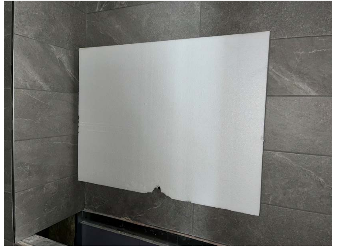
Mirror installation ongoing
