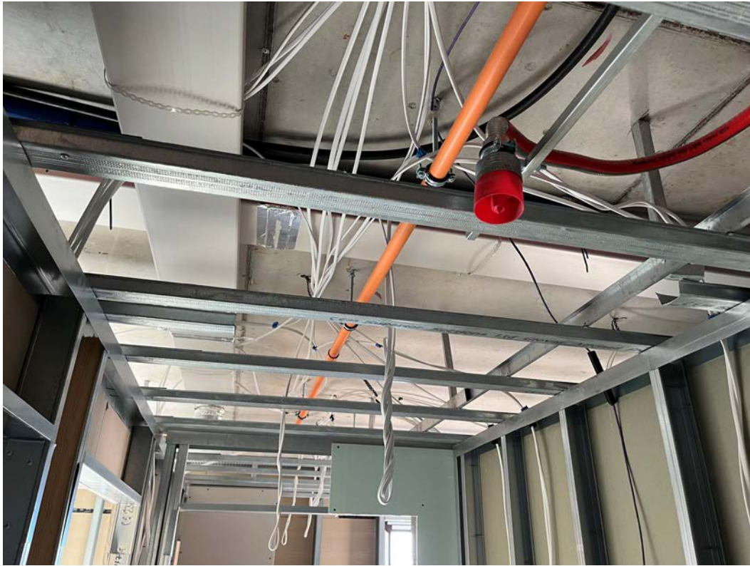
1 st fix electrical installation ongoing
