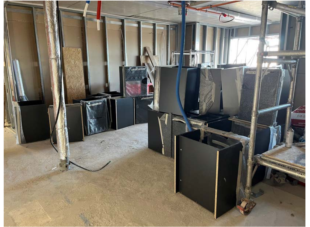
Kitchen units on site
