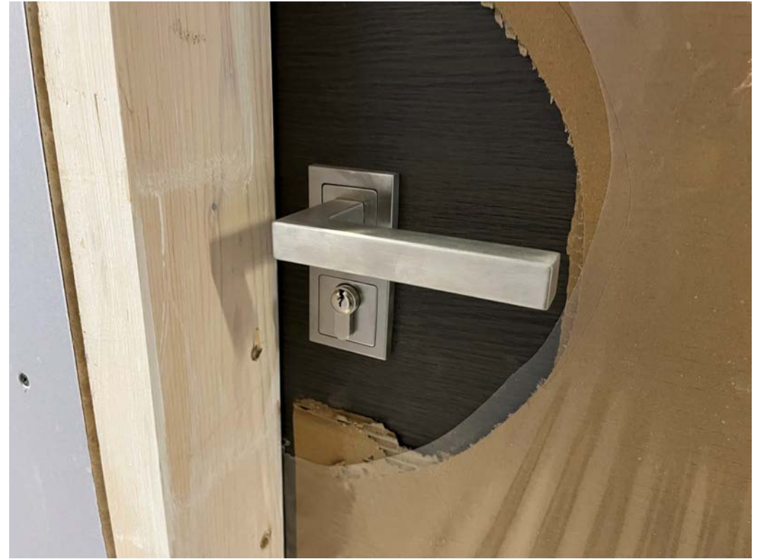
Ironmongery installation ongoing
