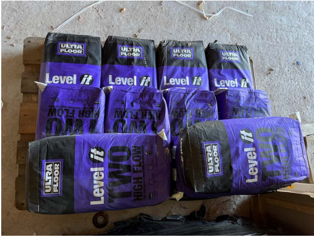
Self-levelling screed on site
