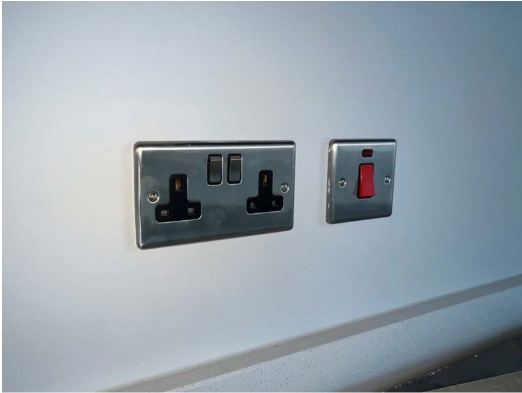
2nd fix electrical installation ongoing
