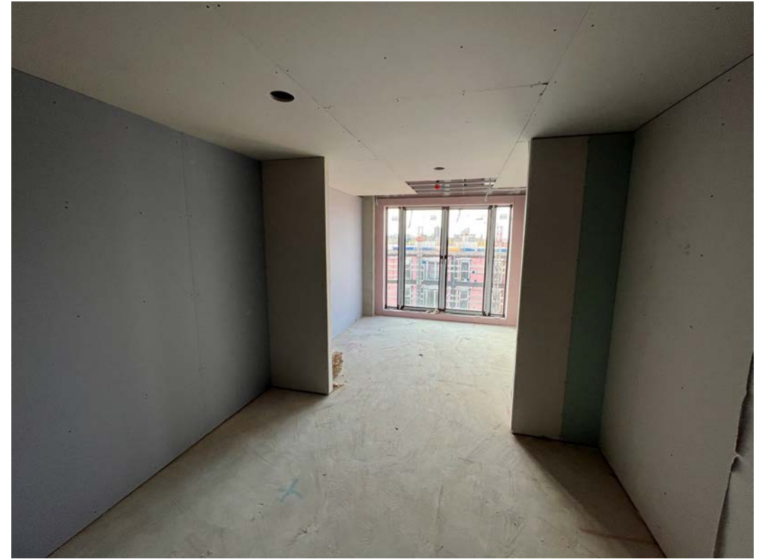
2 nd side boarding of walls and ceilings ongoing
