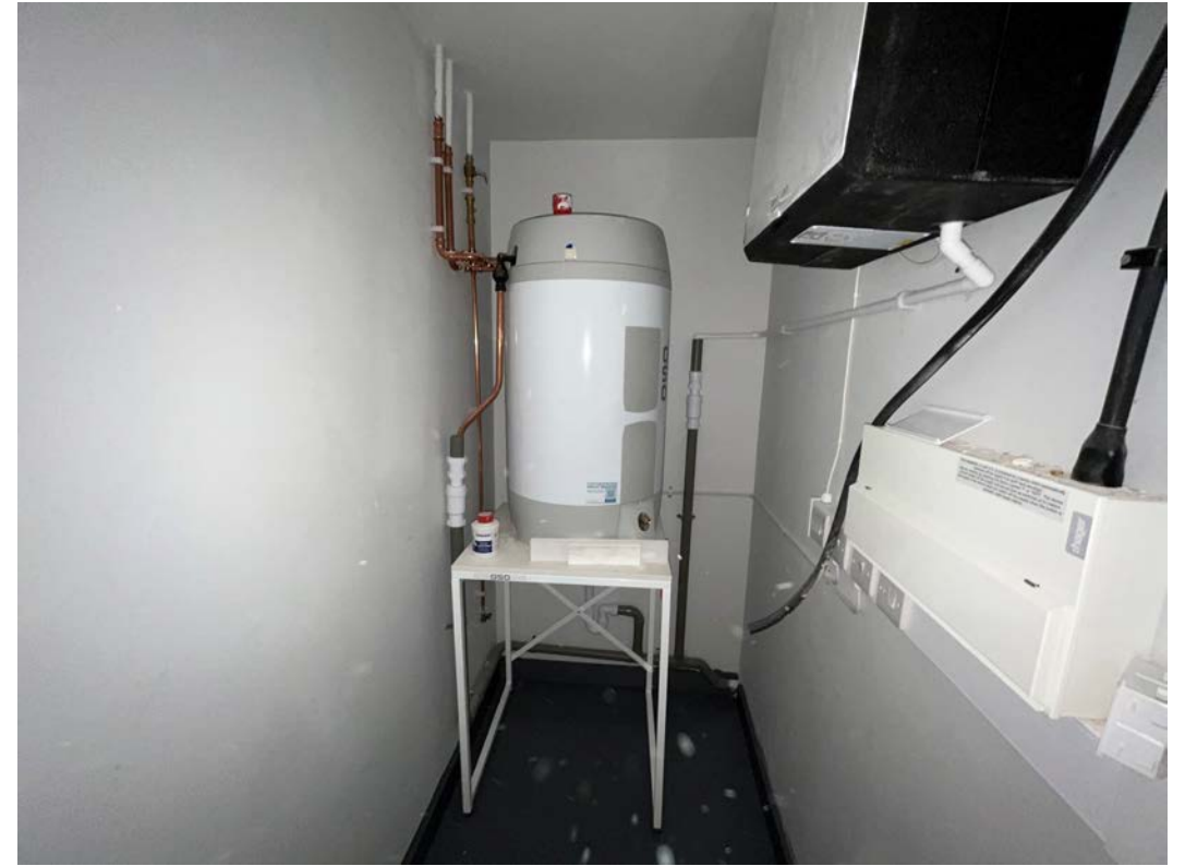
2nd fix mechanical installation ongoing
