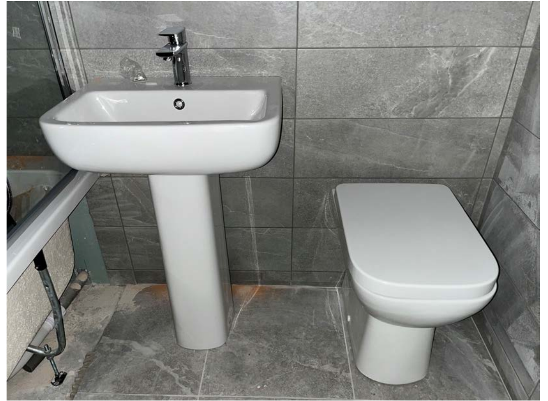
Sanitaryware installation ongoing
