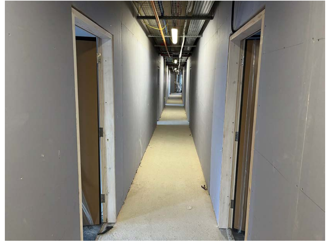
2 nd side boarding of walls and internal joinery ongoing
