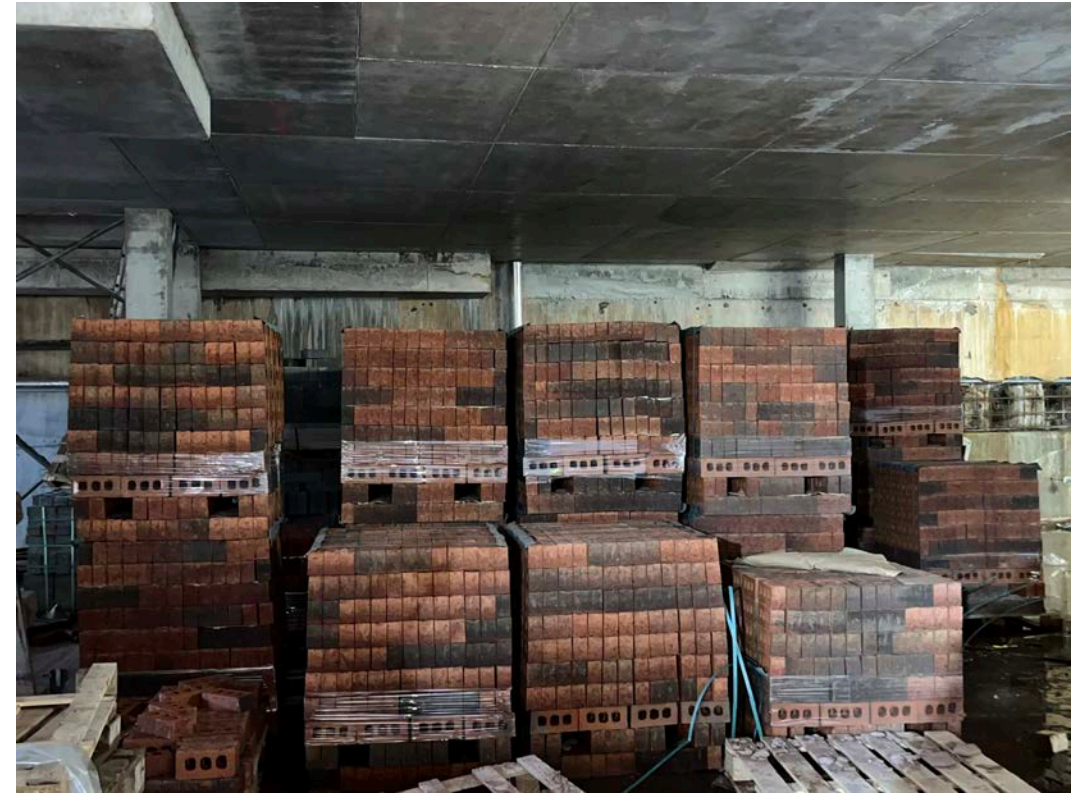
Masonry on site
