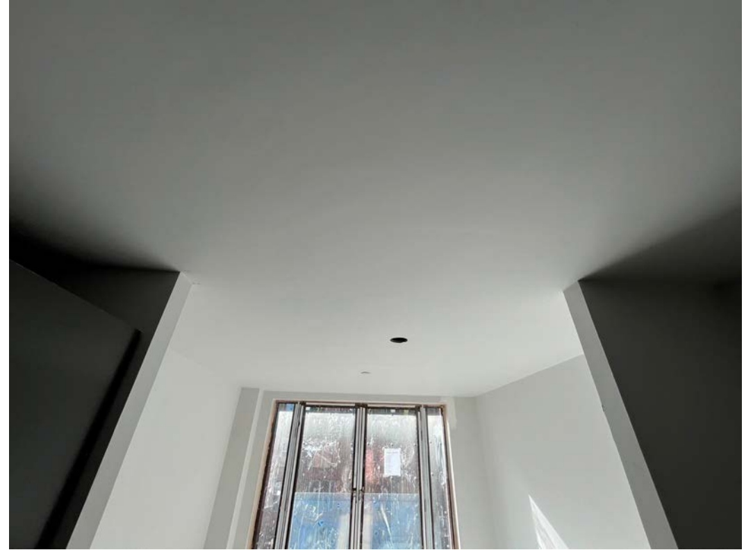
Internal finishes ongoing
