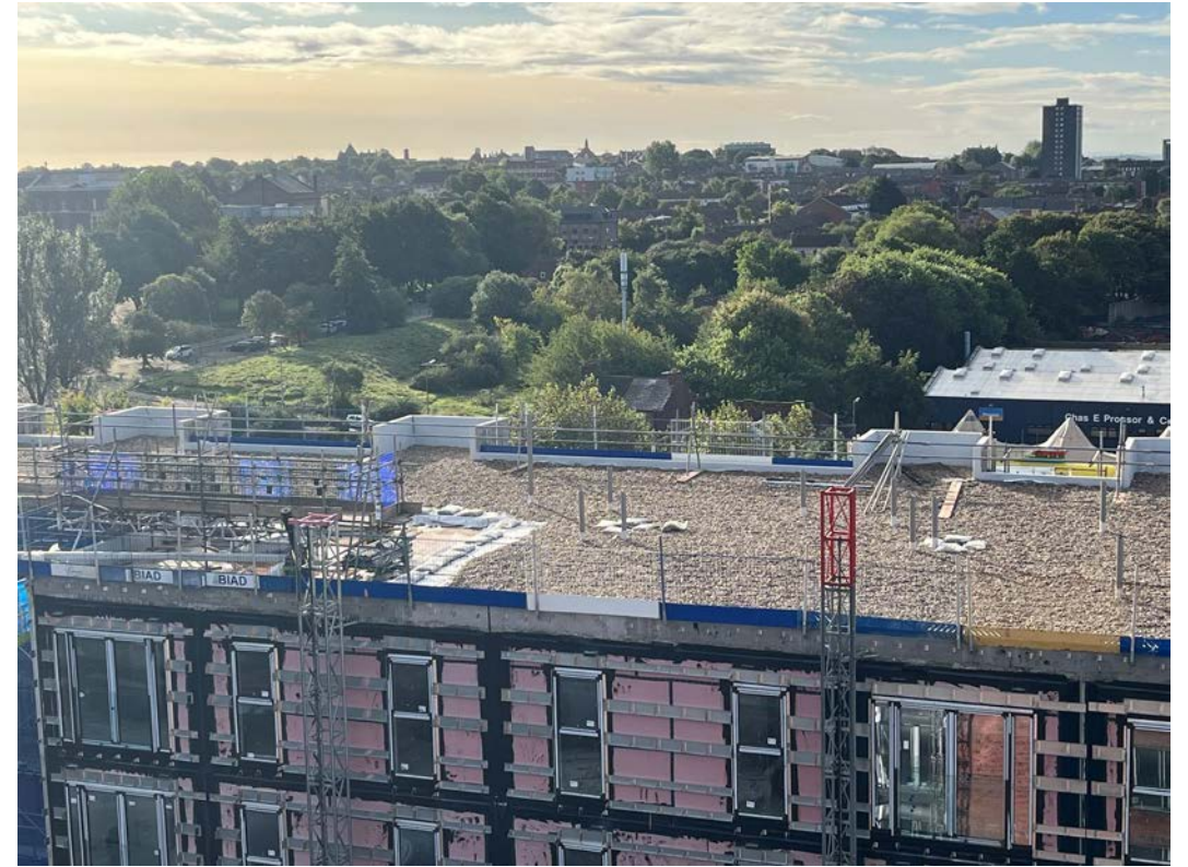
Block D Section A – Flat roof covering ongoing
