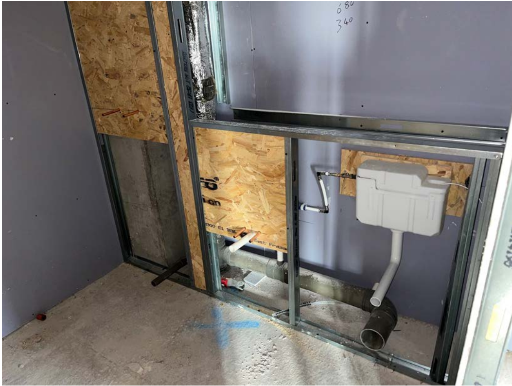
Pan installation and formation IPS ongoing
