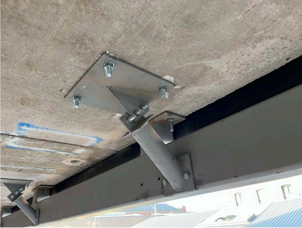
Steel supports installed for curtain wall
