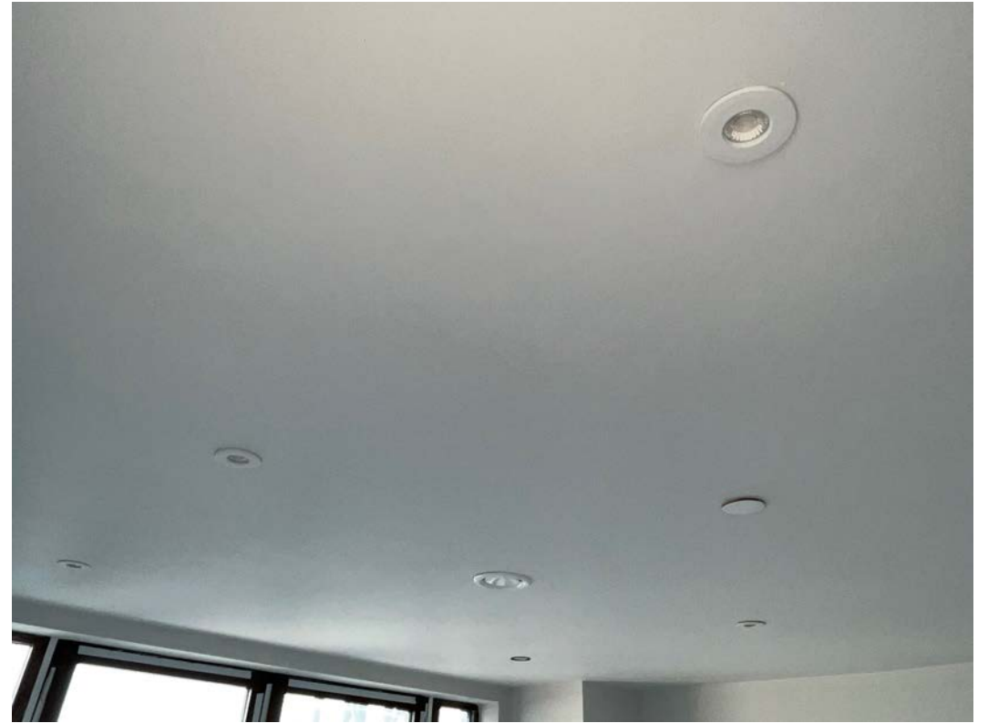
2nd fix electrical installation ongoing
