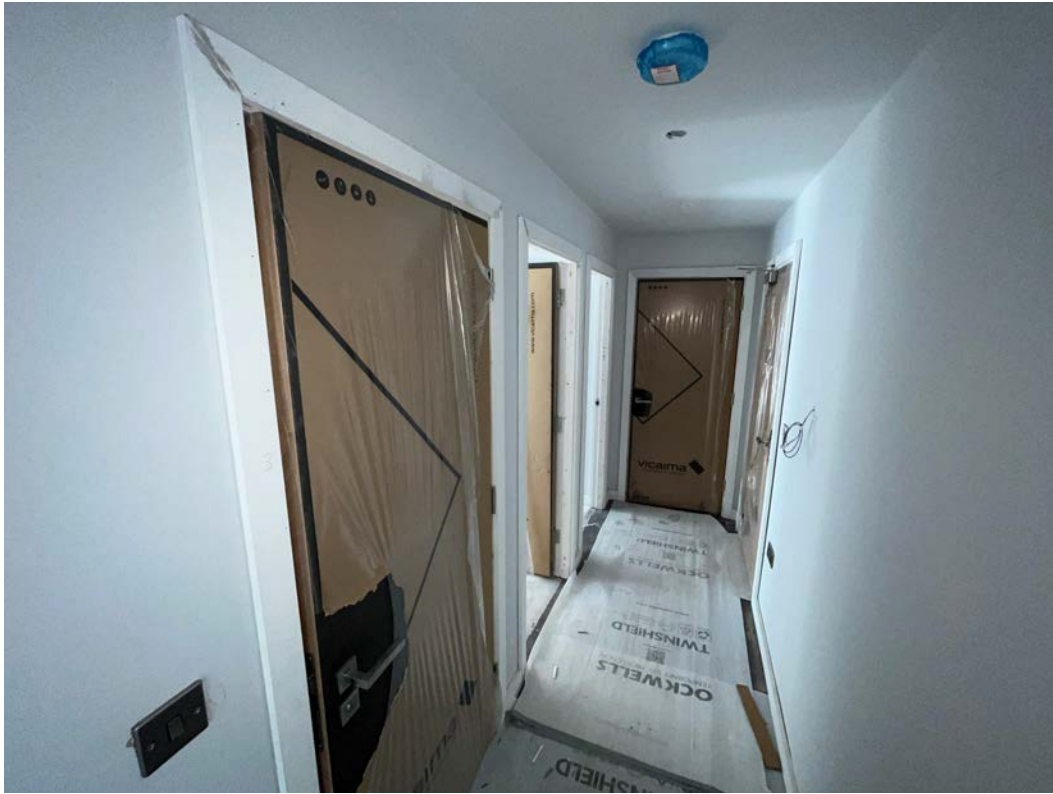
Internal joinery and doors installation ongoing
