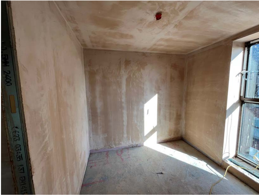
Plaster skim walls and ceiling application ongoing
