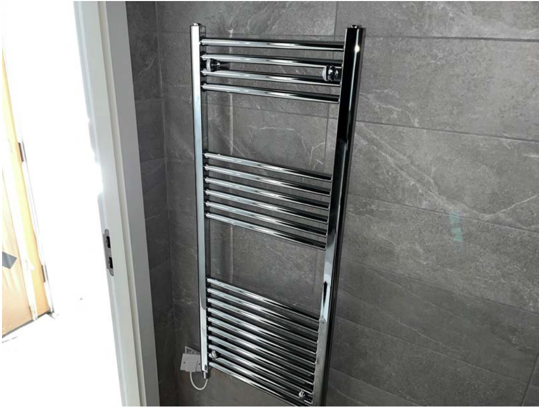
Heated towel rail installation ongoing
