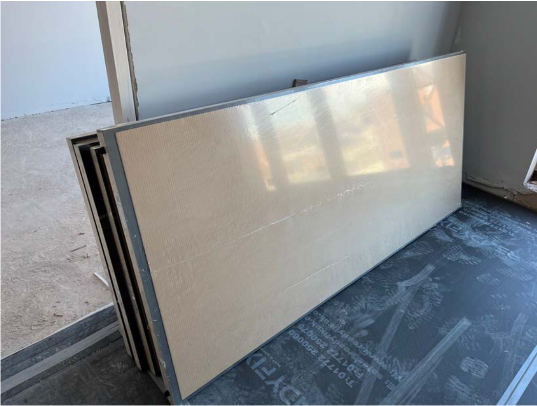
Internal doors on site
