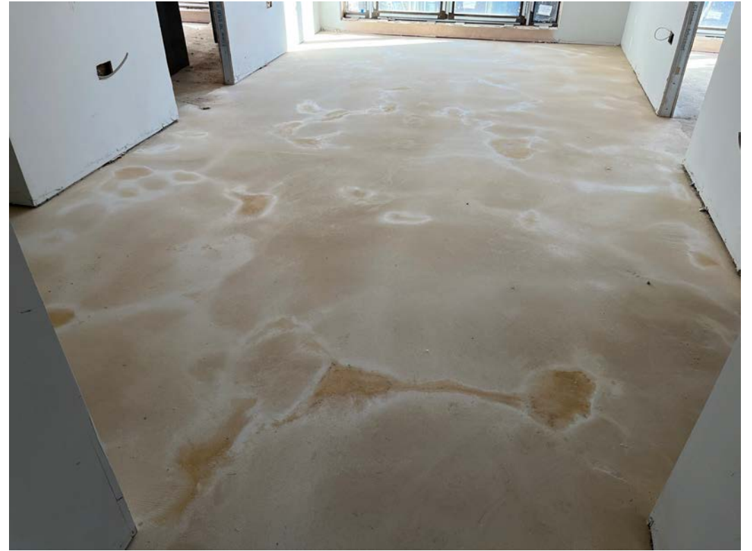
Self-levelling screed application ongoing
