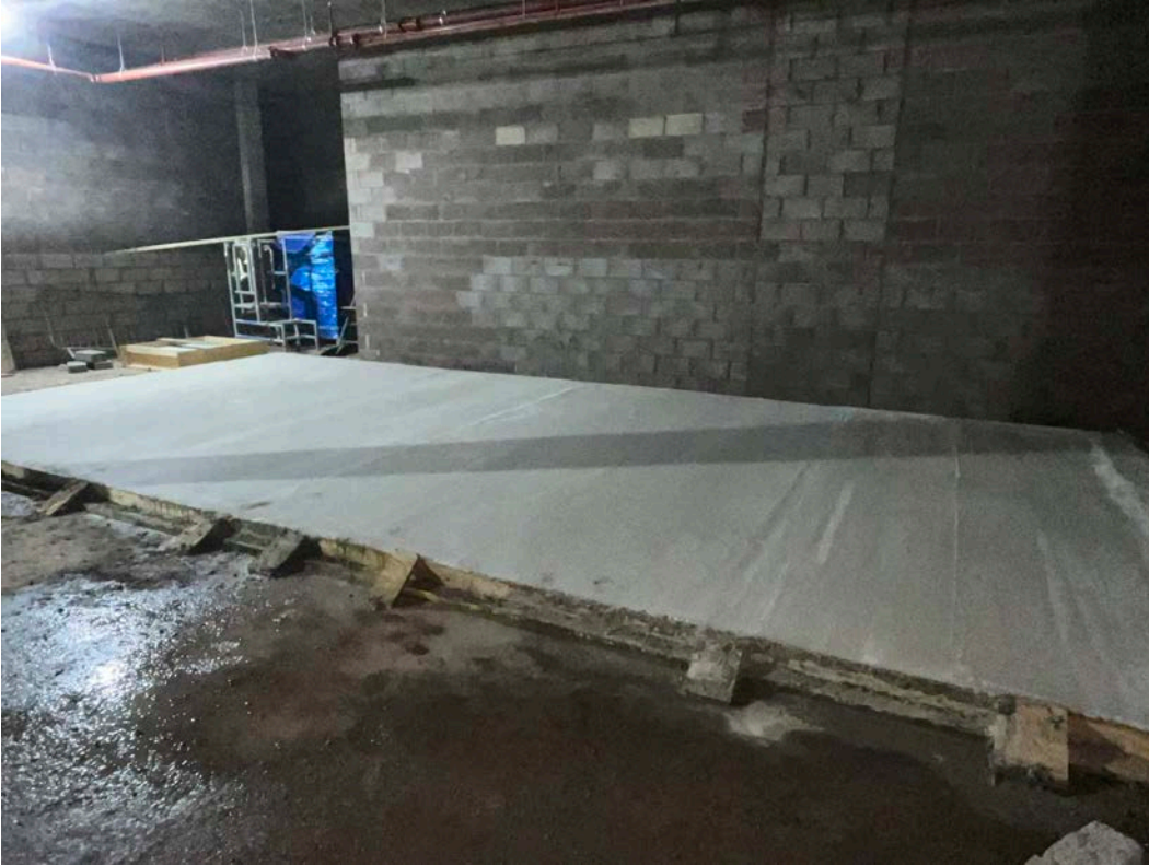
Block D Section A – Concrete slab
