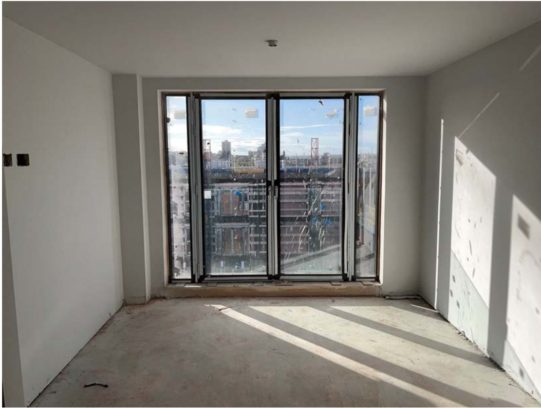
Internal finishes ongoing
