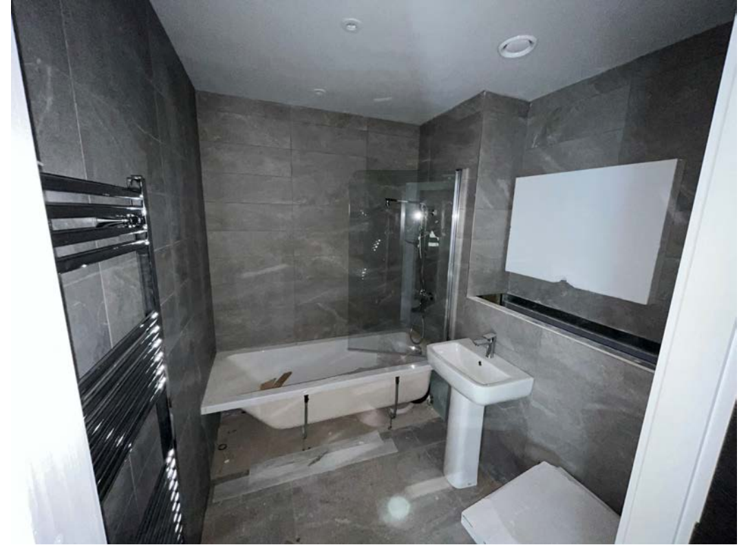
Sanitaryware installation ongoing
