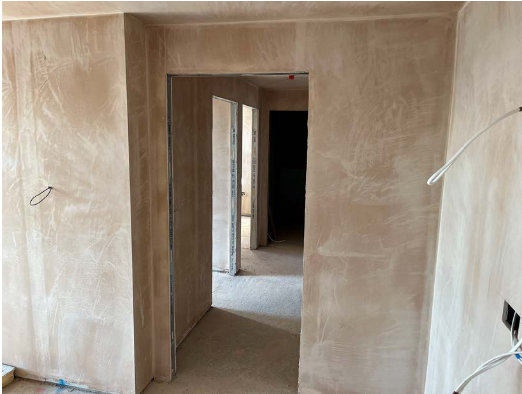
Plaster skim walls and ceiling application ongoing
