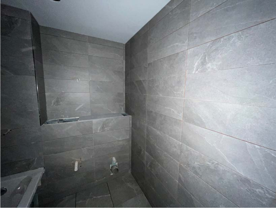
Wall and floor tile installation ongoing
