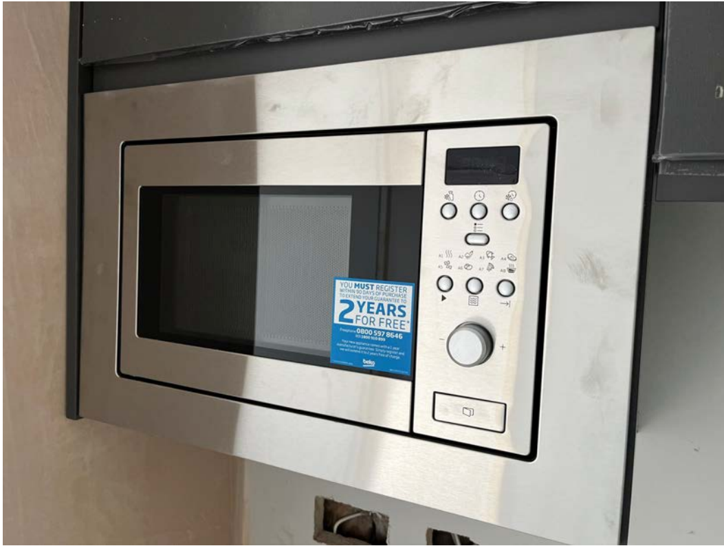
Installation of kitchen appliances ongoing
