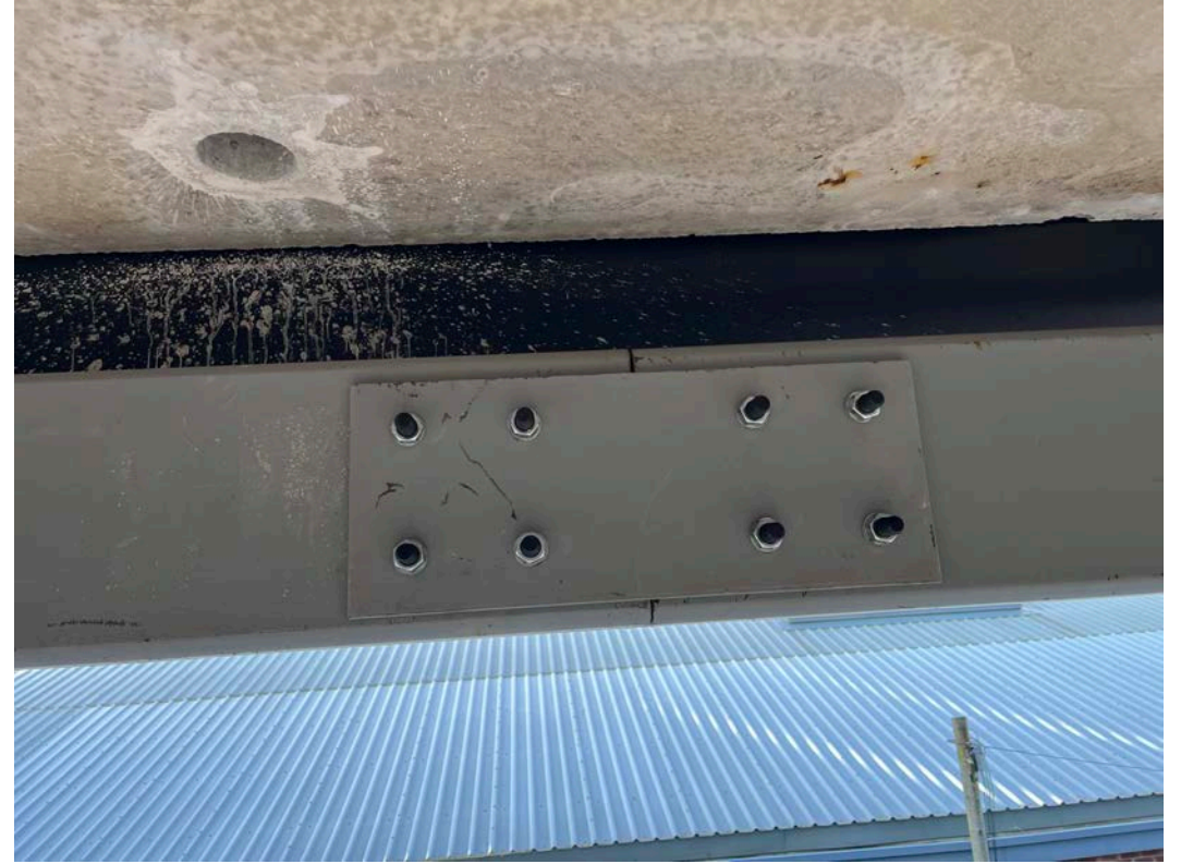
Steel supports installed for curtain wall
