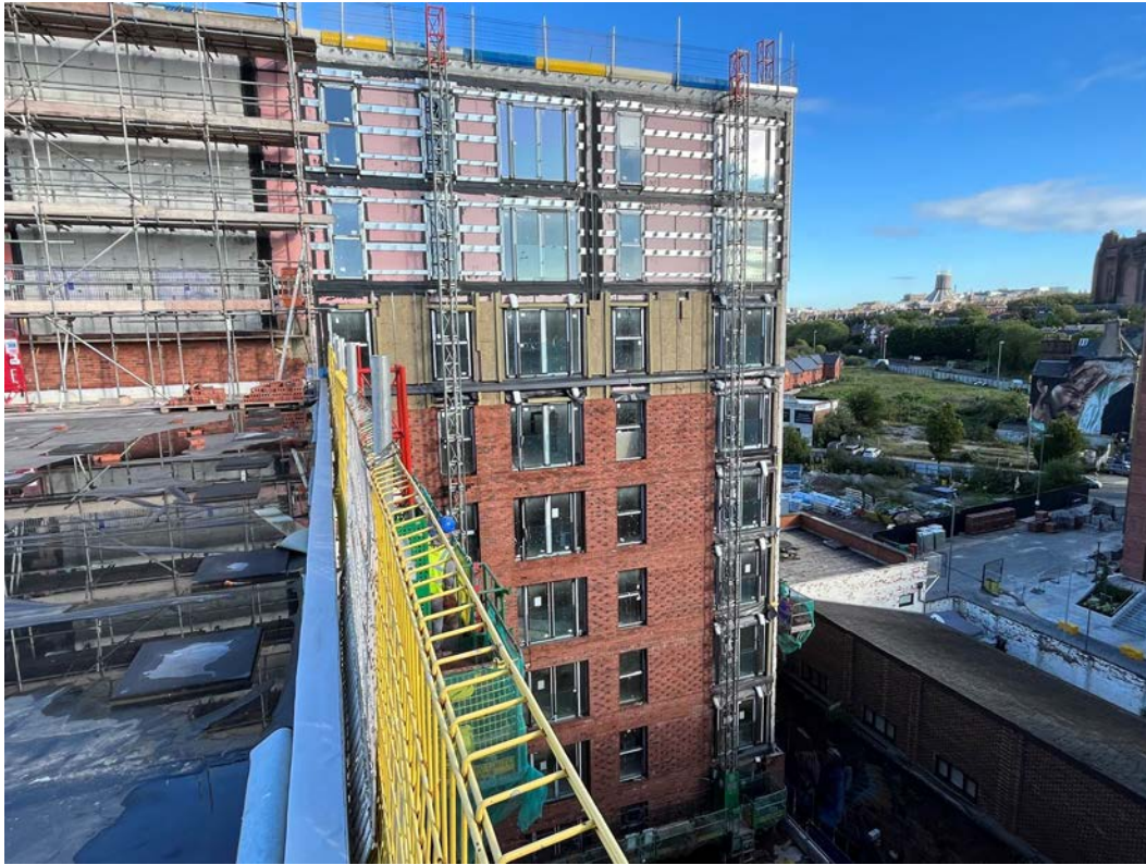
Block D Section A – External insulation and brickwork ongoing
