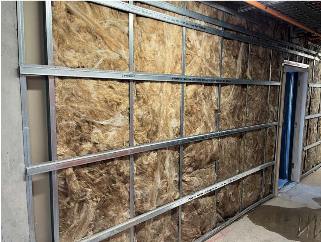
1 st side boarding of walls and insulation installation ongoing
