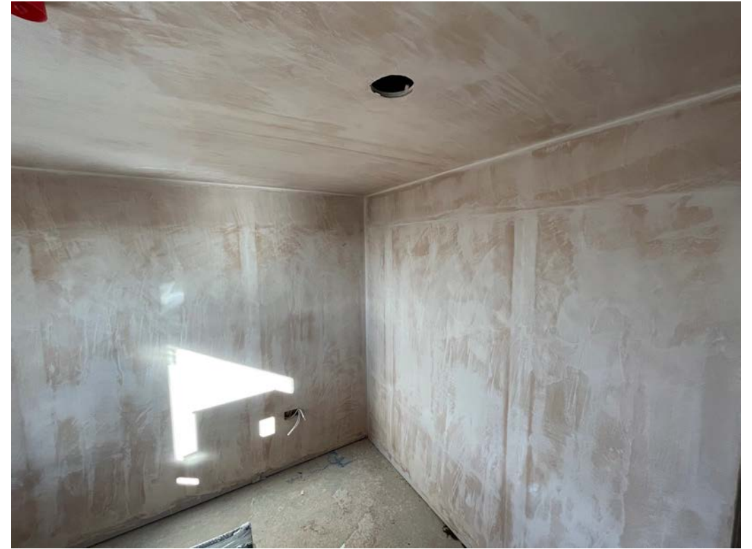
Plaster skim walls and ceiling application ongoing
