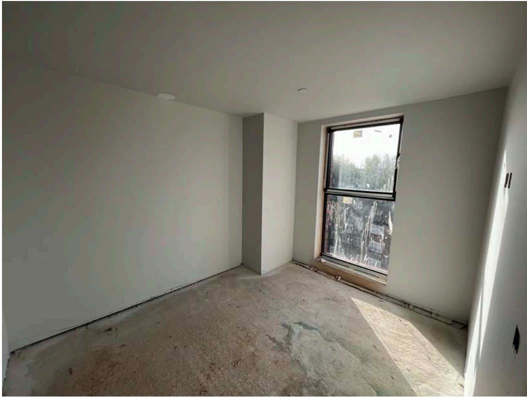
Internal finishes ongoing
