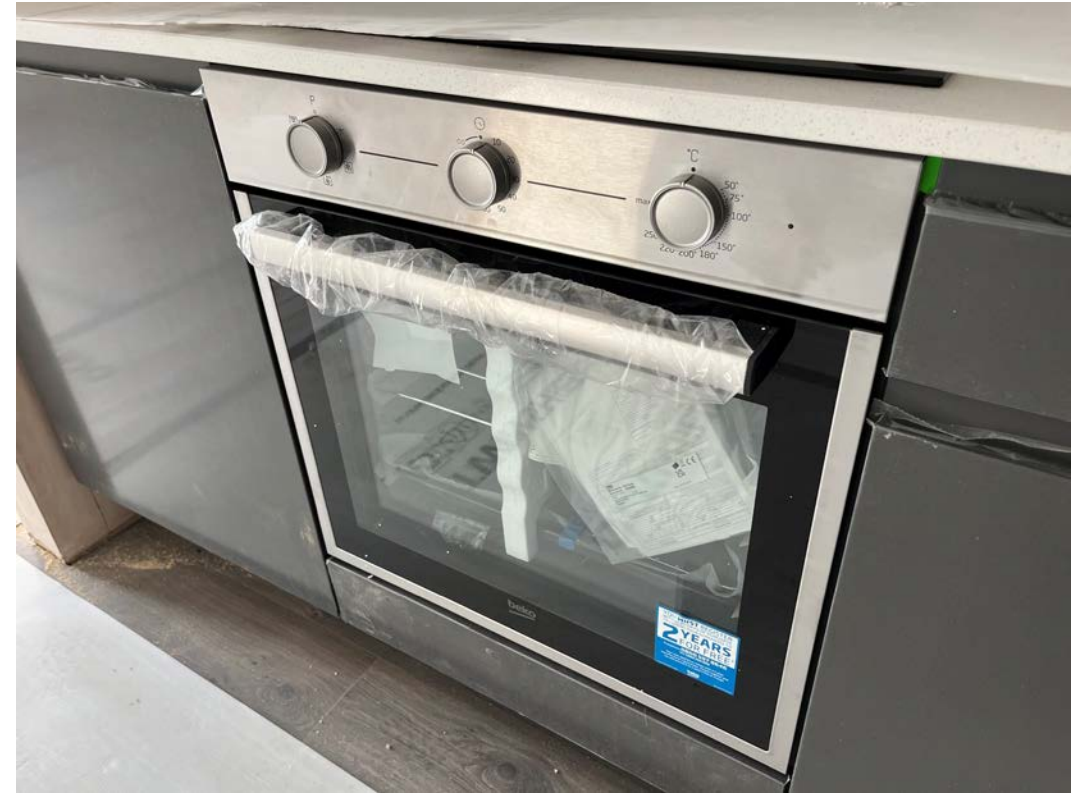
Installation of kitchen appliances ongoing
