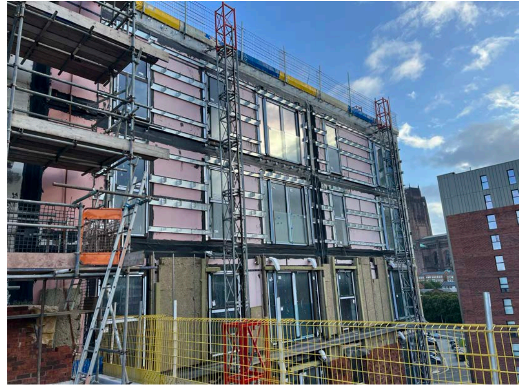
Block D Section A – Cladding brackets installed
