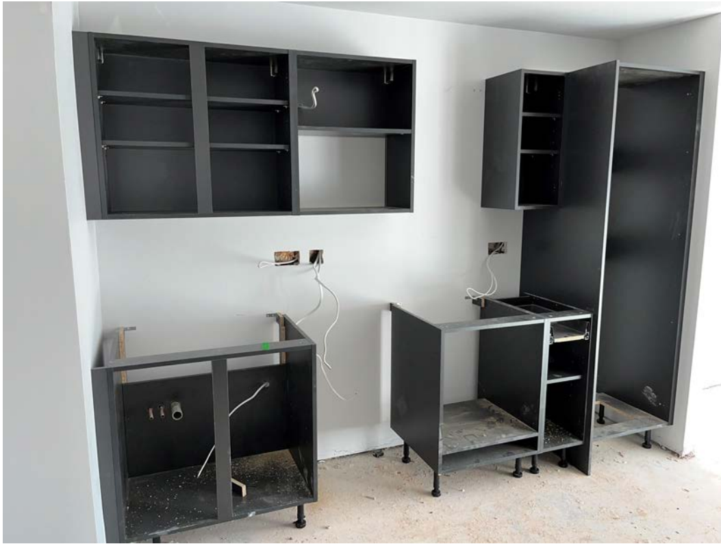
Installation of kitchen units and worktops ongoing
