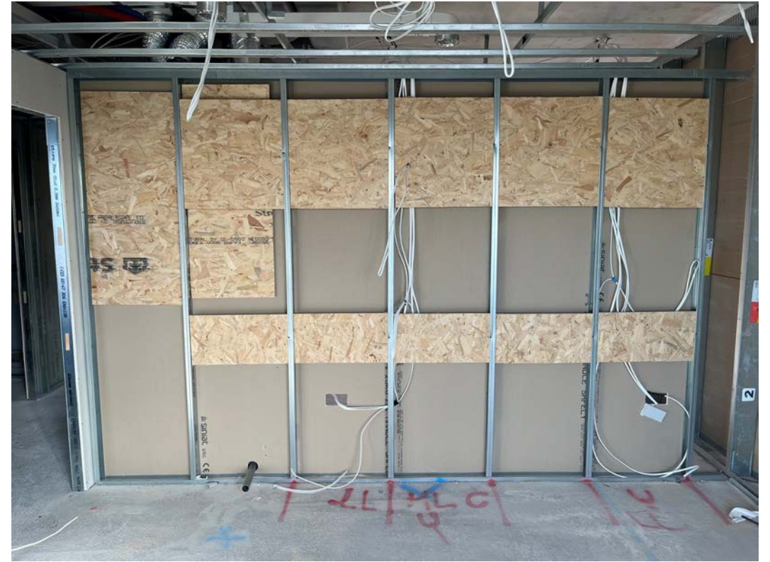
Pattress installation ongoing
