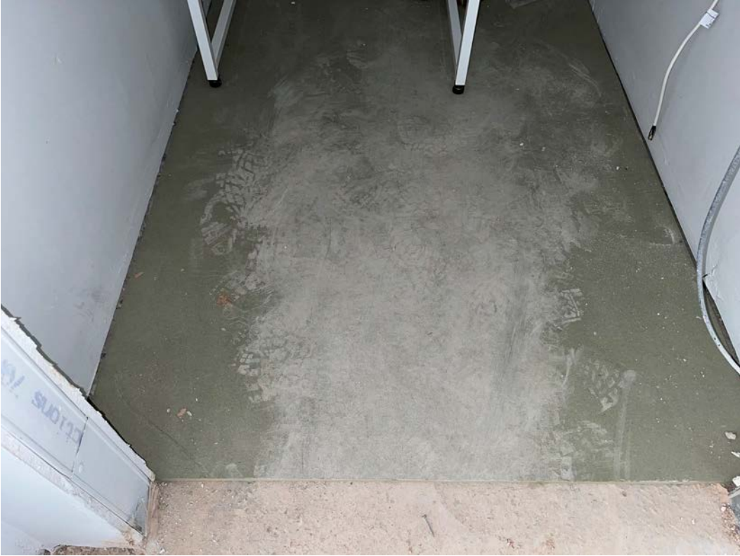
Cylinder cupboard floor installation ongoing
