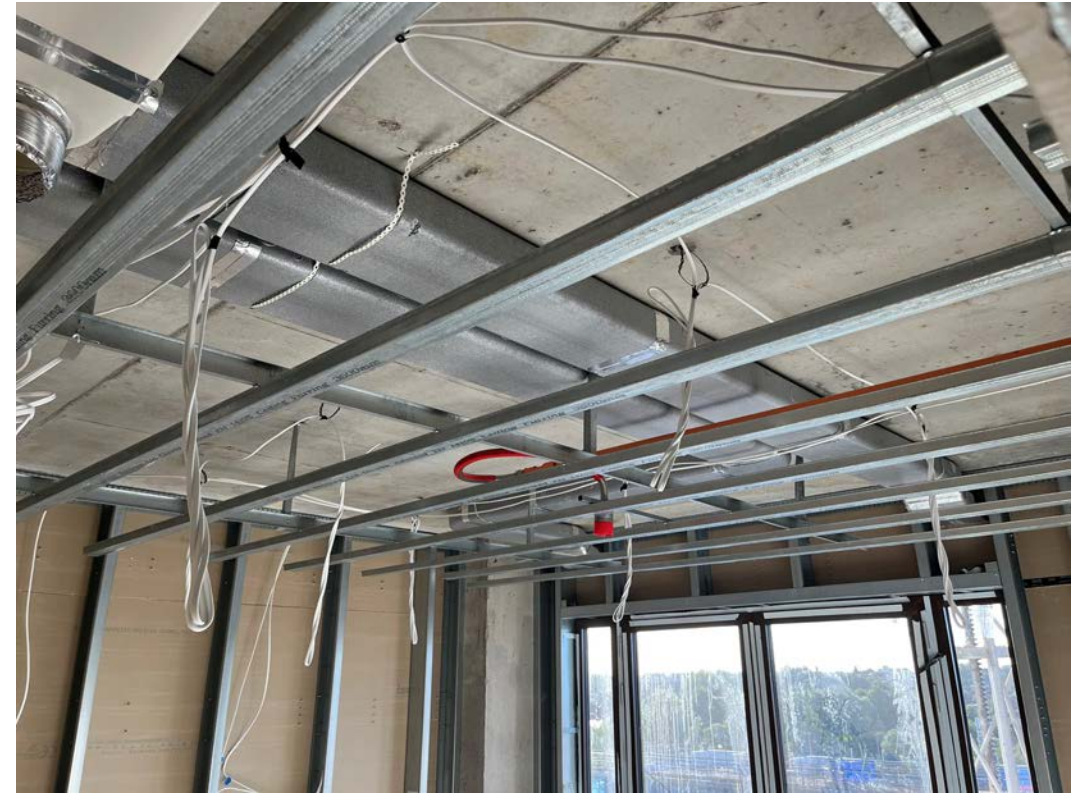
Metal ceiling grid installation ongoing
