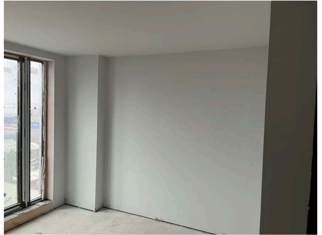
Internal finishes ongoing
