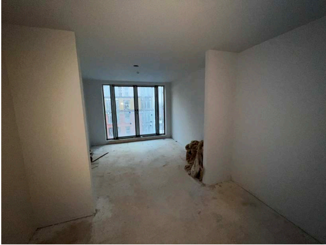
Internal finishes ongoing
