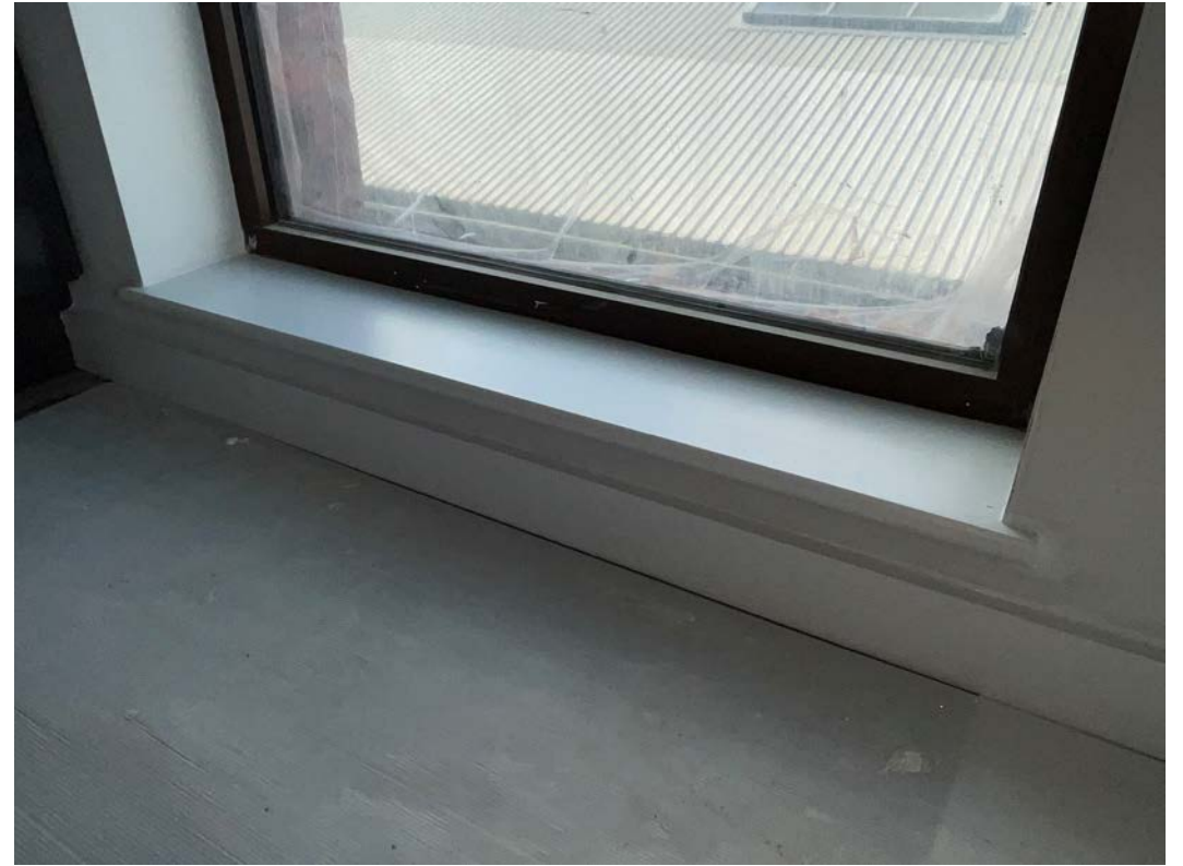
Window and skirting boards installation ongoing
