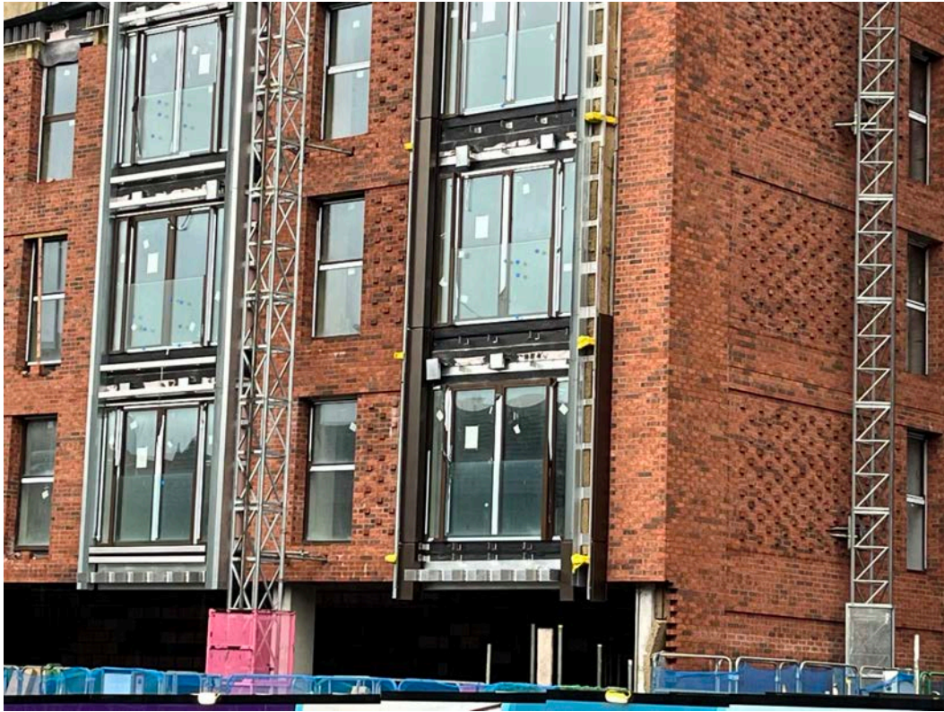
Block D Section B – Installation of external cladding ongoing
