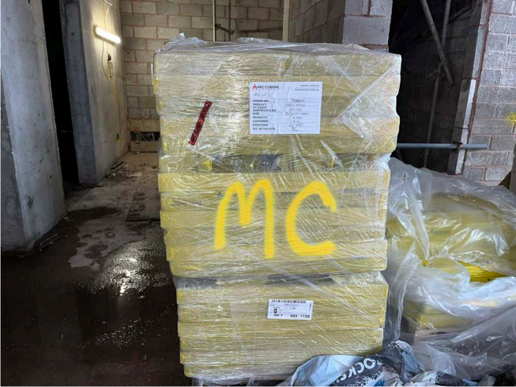
Cavity barrier on site
