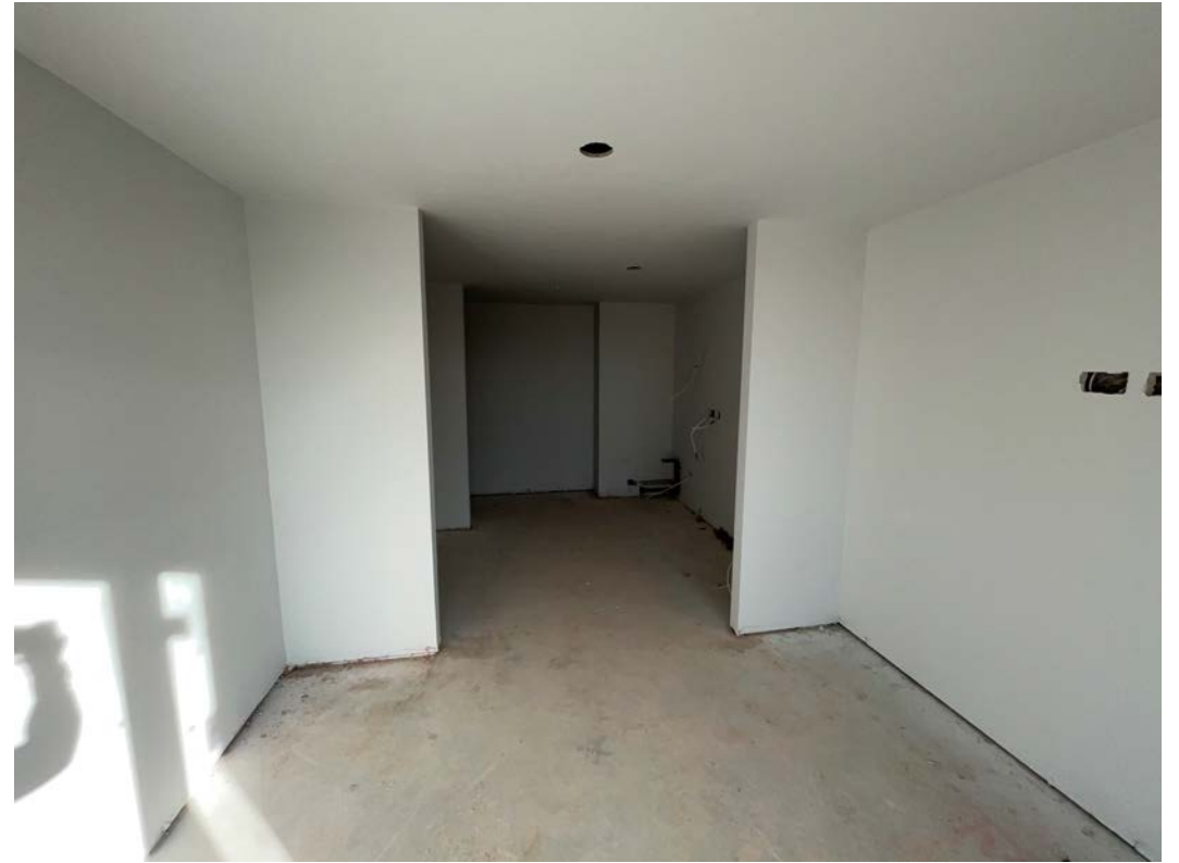
Internal finishes ongoing
