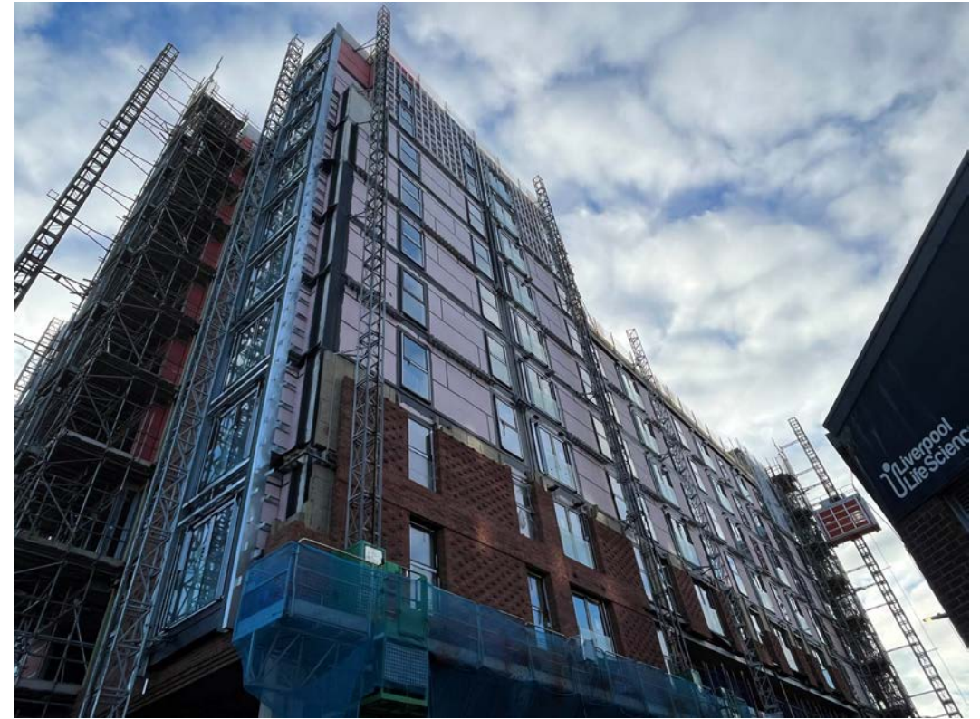
Block D Section A and C – External insulation and brickwork ongoing
