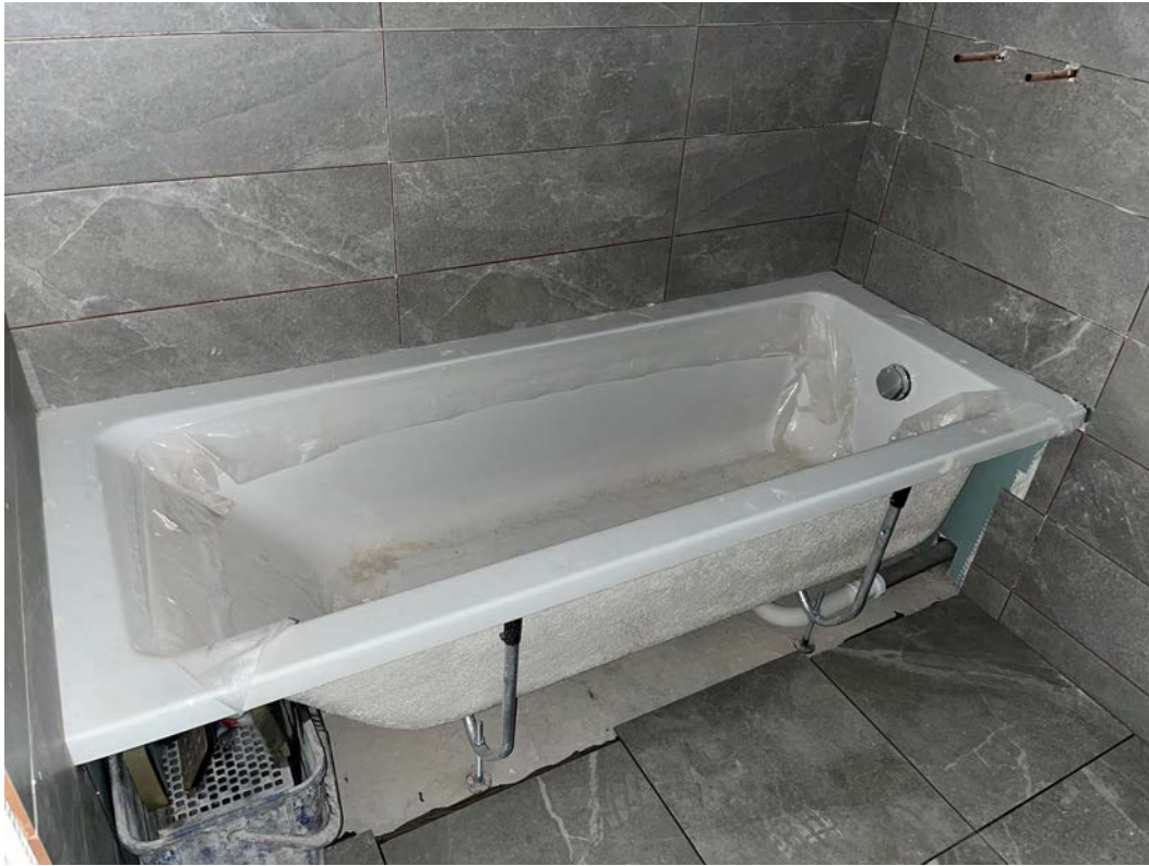
Sanitaryware installation ongoing
