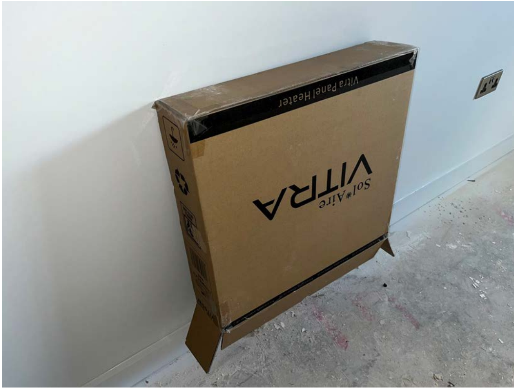
Electrical wall heater installation ongoing
