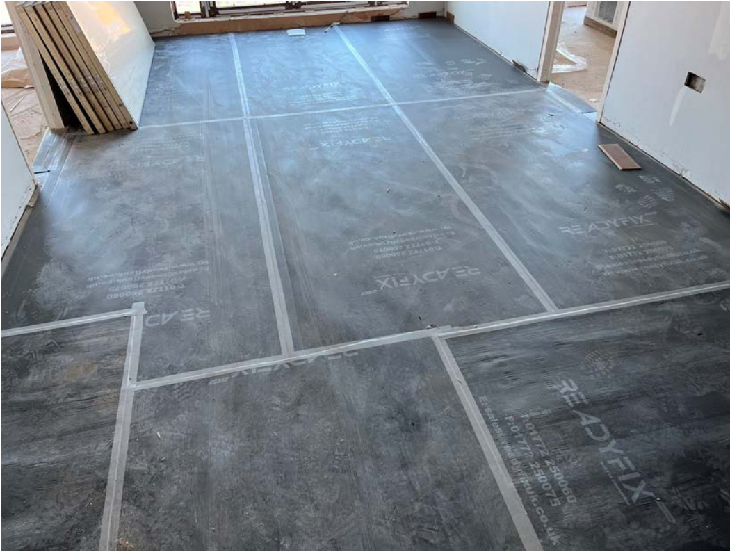
Laminate flooring and protection installation ongoing
