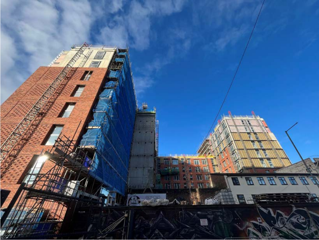
Block D Section B, C & A – Viewed from Crump Street
