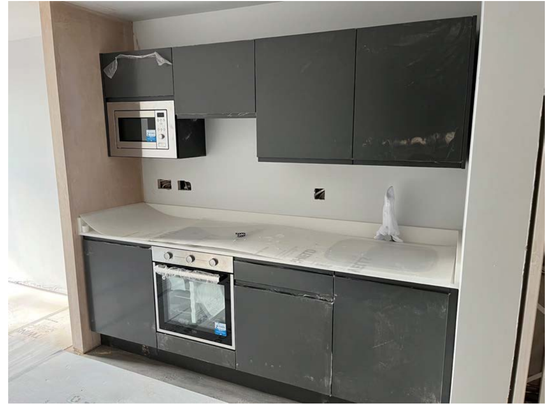
Installation of kitchen units and appliances ongoing
