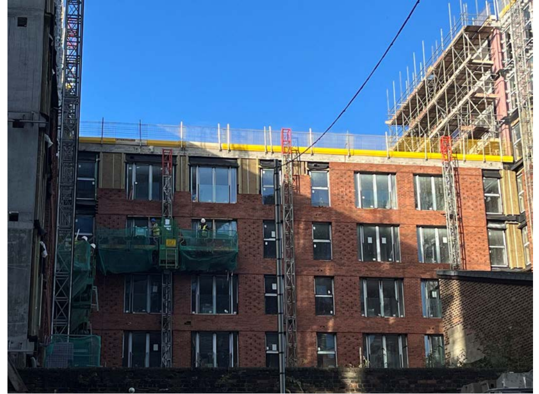
Block D Section C – Viewed from Crump Street
