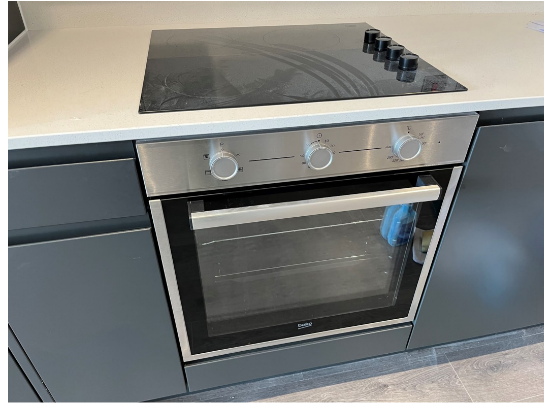
Installation of kitchen appliances ongoing
