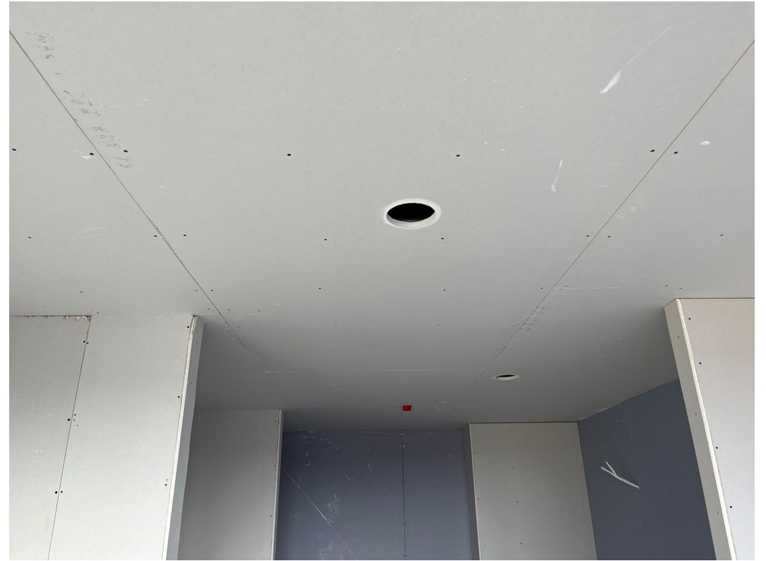
2 nd side boarding of ceilings ongoing
