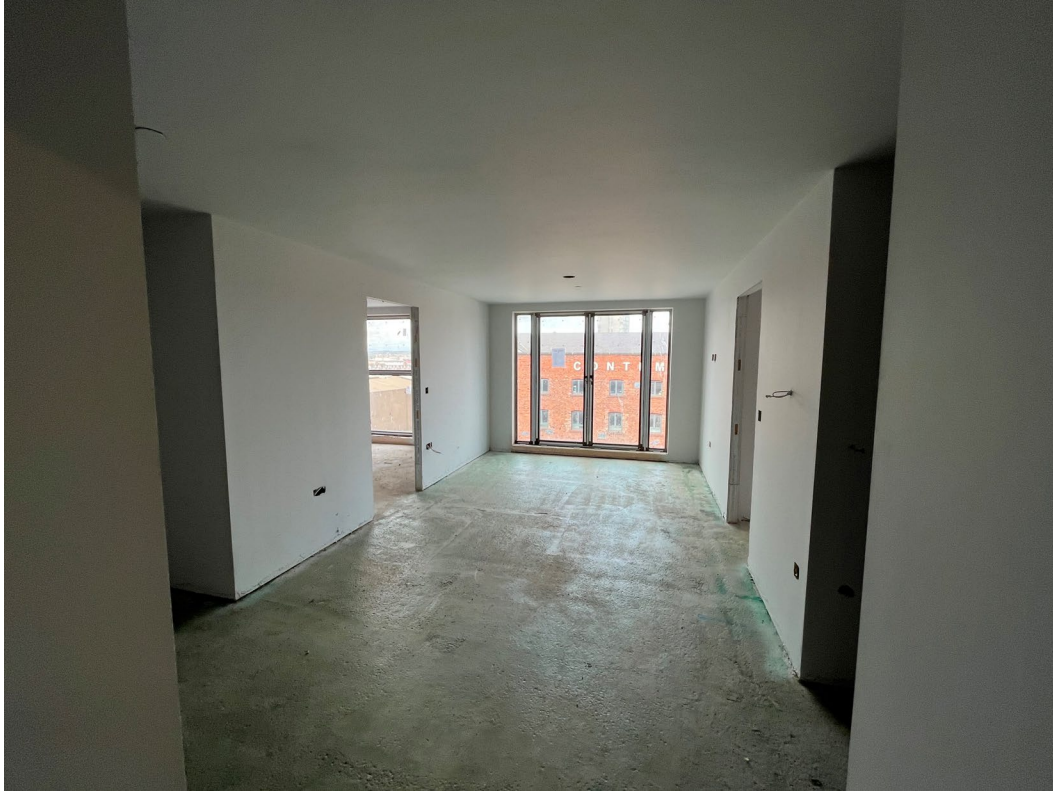
Internal finishes ongoing
