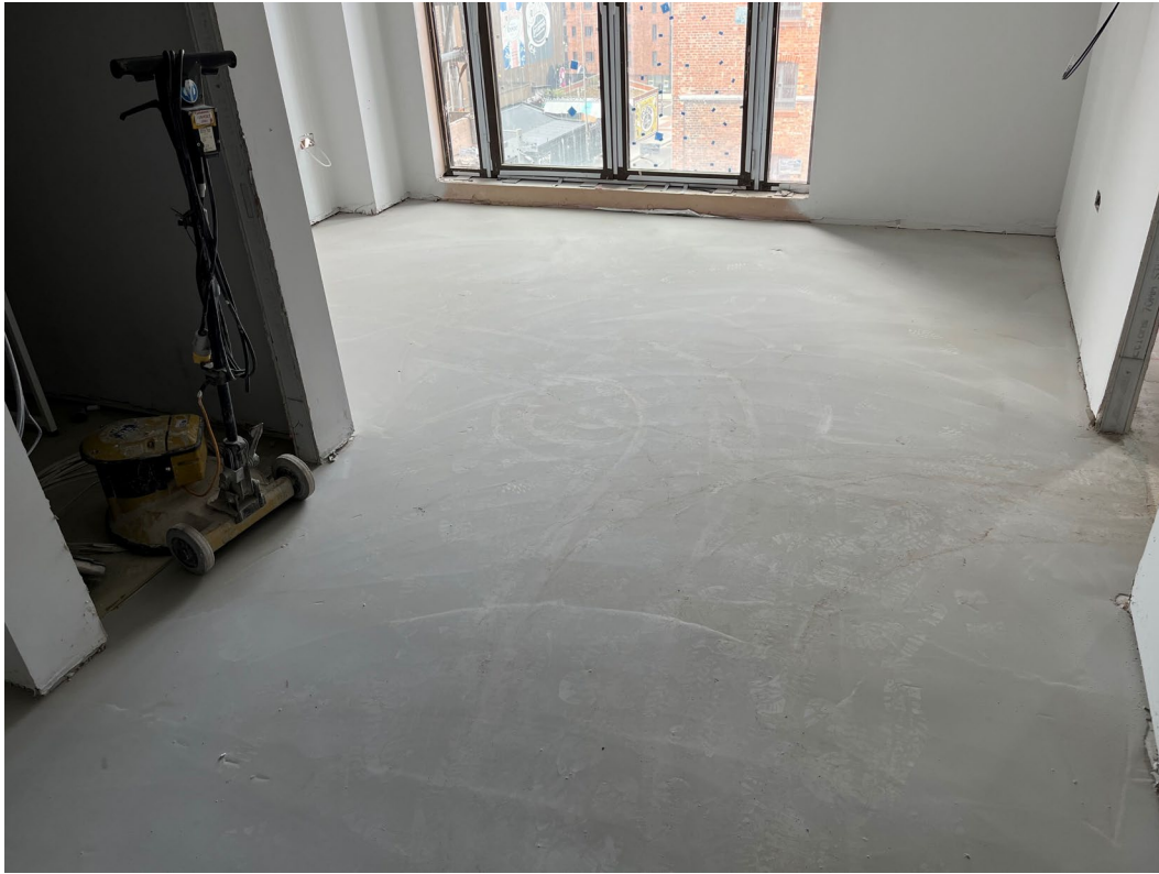
Self-levelling screed application ongoing
