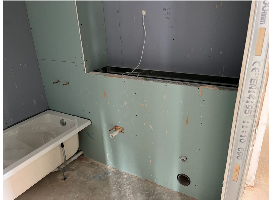
2 nd side boarding of IPS ongoing
