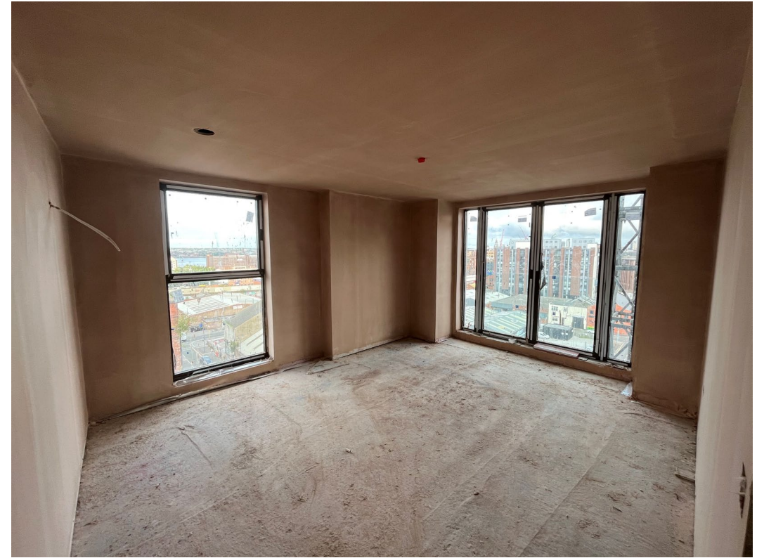
Plaster skim walls and ceiling application ongoing
