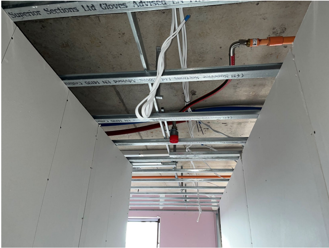
1 st fix electrical installation ongoing
