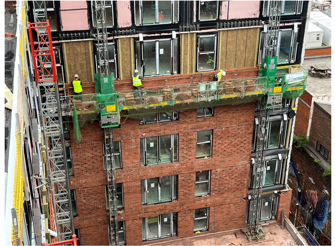
Block D Section A – External insulation and brickwork installation
