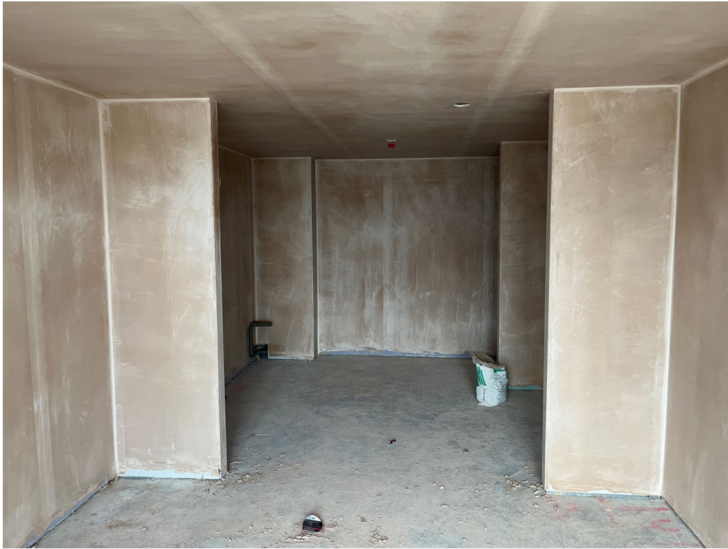
Plaster skim walls and ceiling application ongoing
