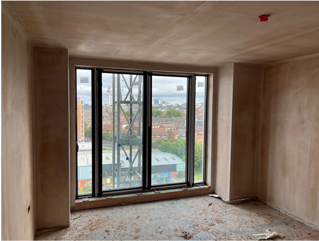
Plaster skim walls and ceiling application ongoing
