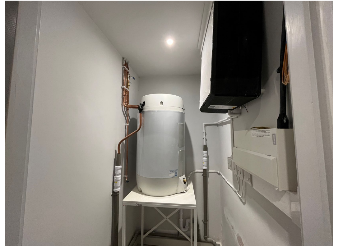
2 nd fix mechanical installation ongoing
