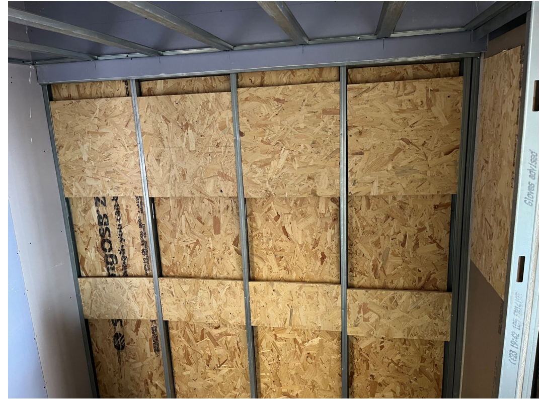
Pattress installation ongoing
