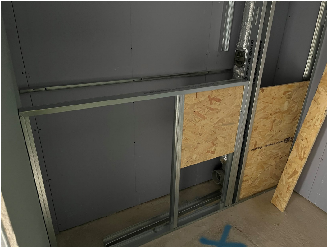
Partness installation and formation IPS ongoing
