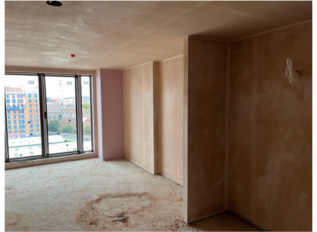
Plaster skim walls and ceiling application ongoing
