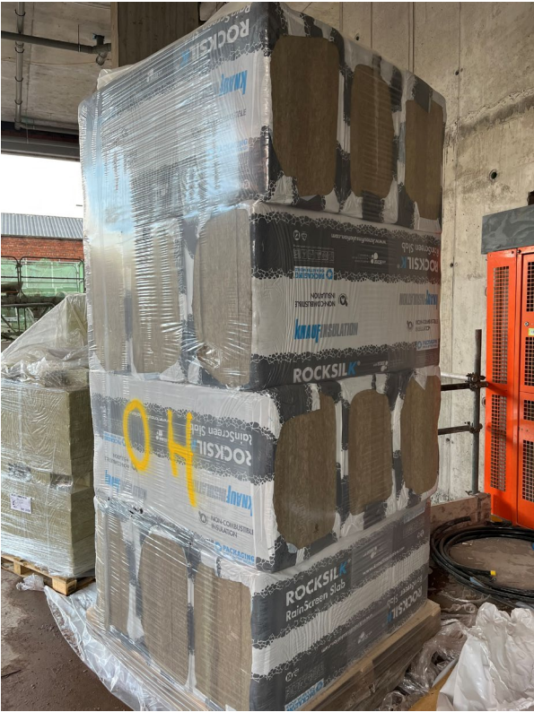
Cavity wall insulation on site
