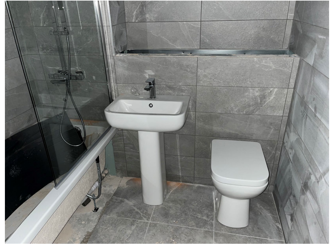
Sanitaryware installation ongoing
