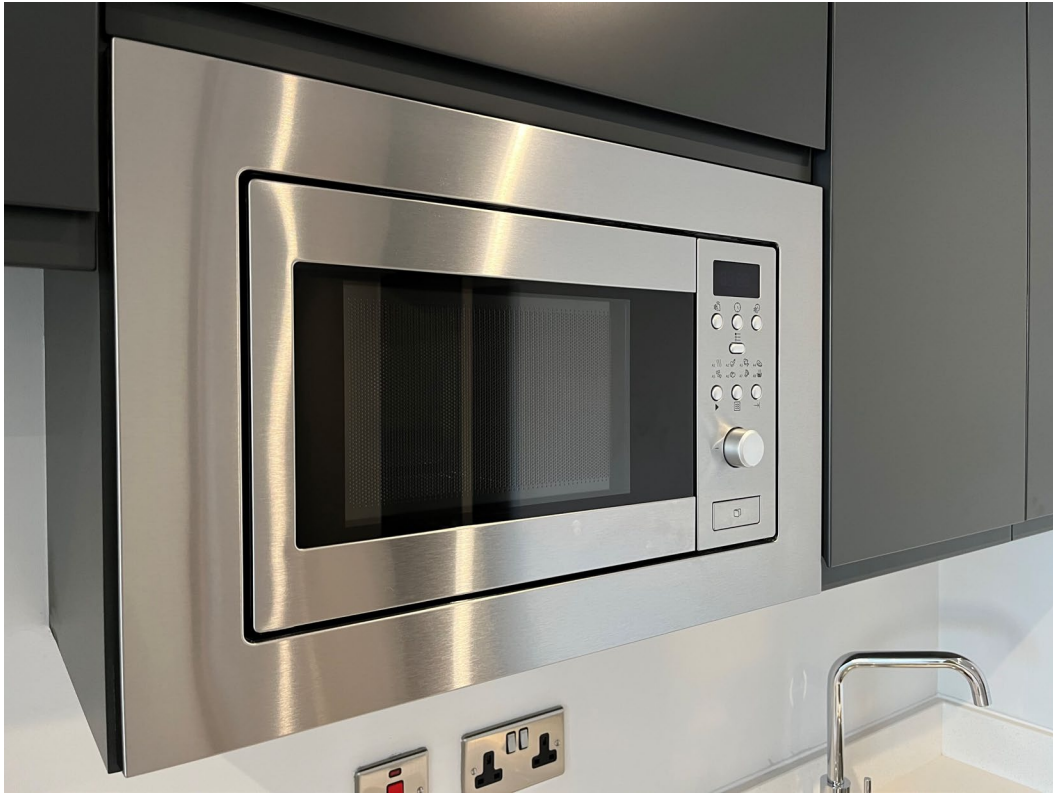
Installation of kitchen appliances ongoing
