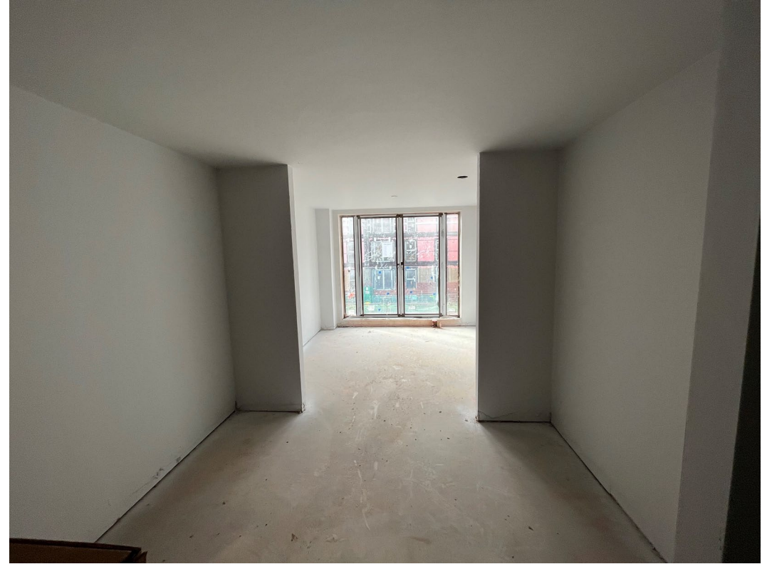
Internal finishes ongoing
