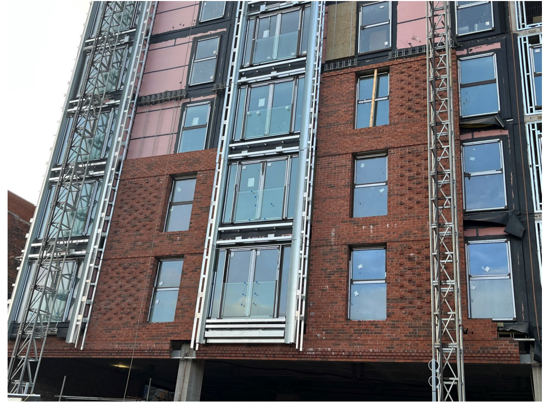
Block D Section A – Masonry supports and external brickwork ongoing
