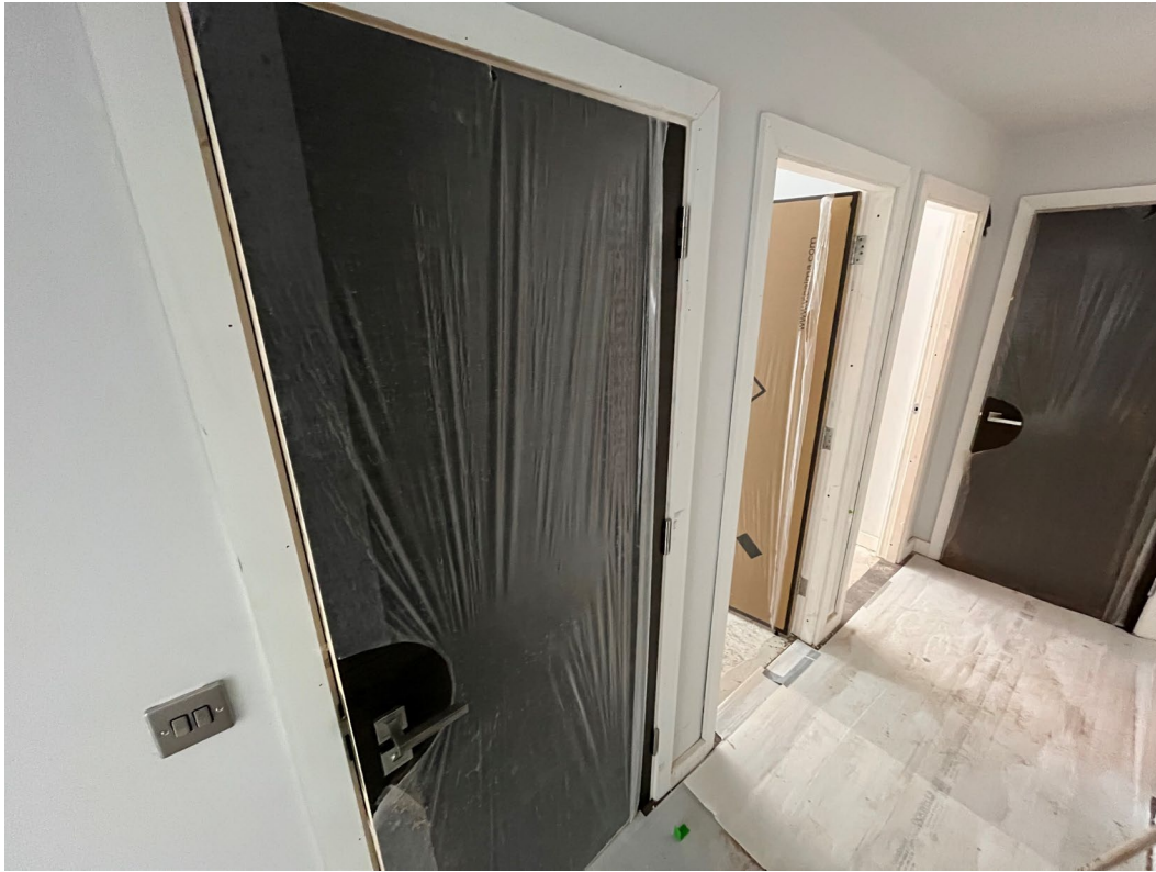
Internal joinery and doors installation ongoing
