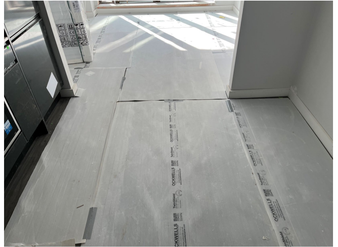
Laminate flooring installation and protection ongoing
