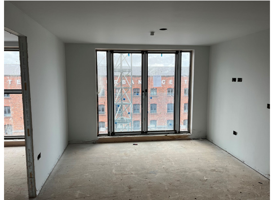
Walls and ceiling mistcoat application
