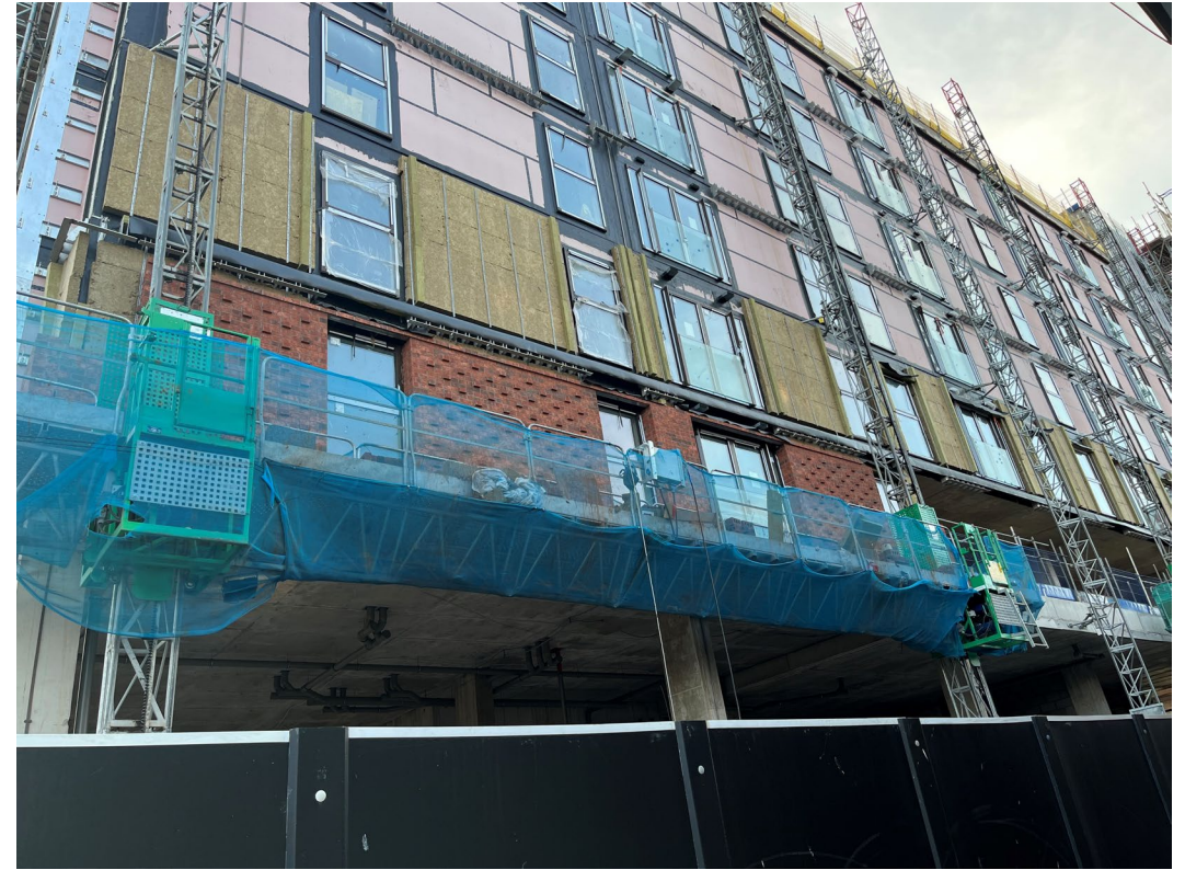
Block D Section A and C – External insulation and brickwork installation
