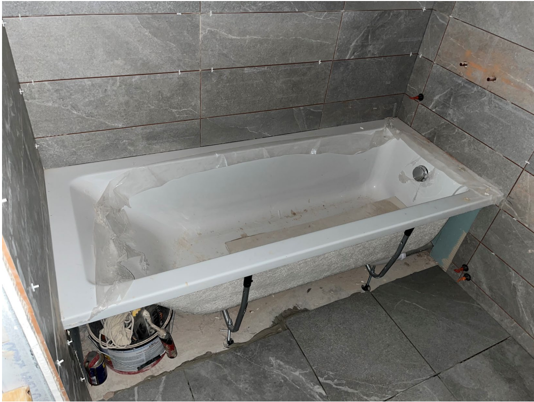
Sanitaryware installation ongoing
