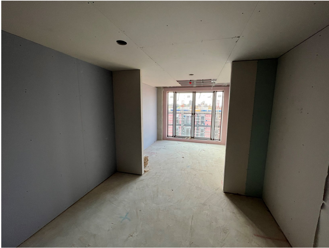
2 nd side boarding of walls ongoing
