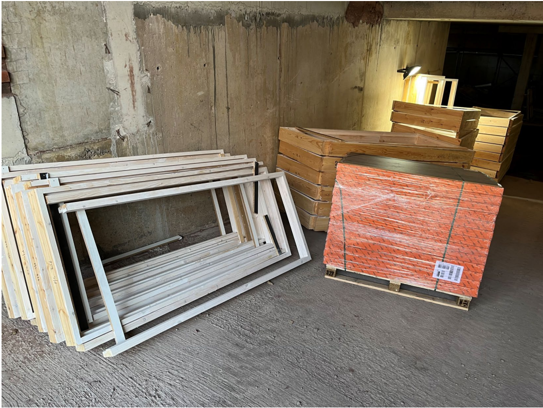
Door frames and laminate flooring on site
