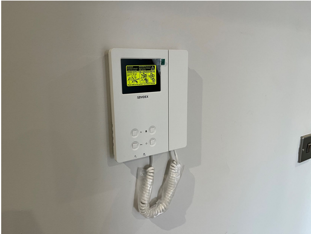
Intercom installation ongoing
