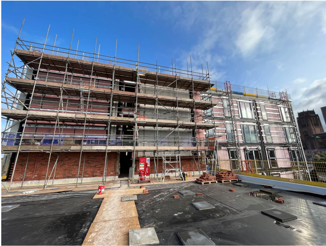
Block D Section A – External brickwork and insulation installation
