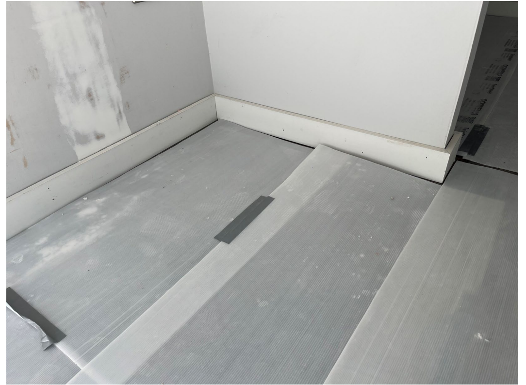
Timber skirting board installation ongoing
