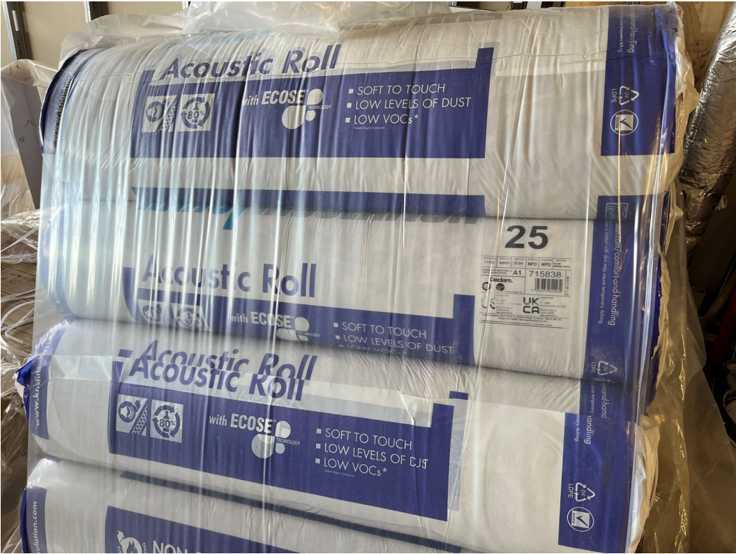
Internal partition insulation on site
