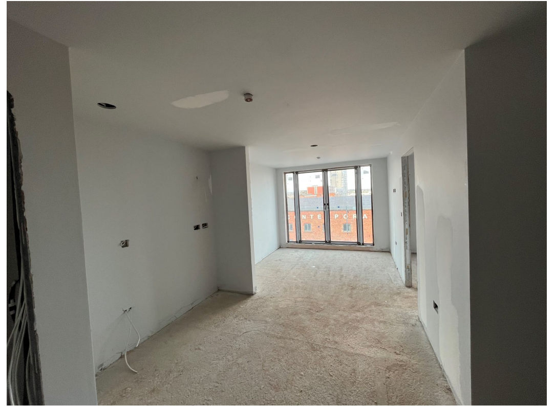
Internal finishes ongoing
