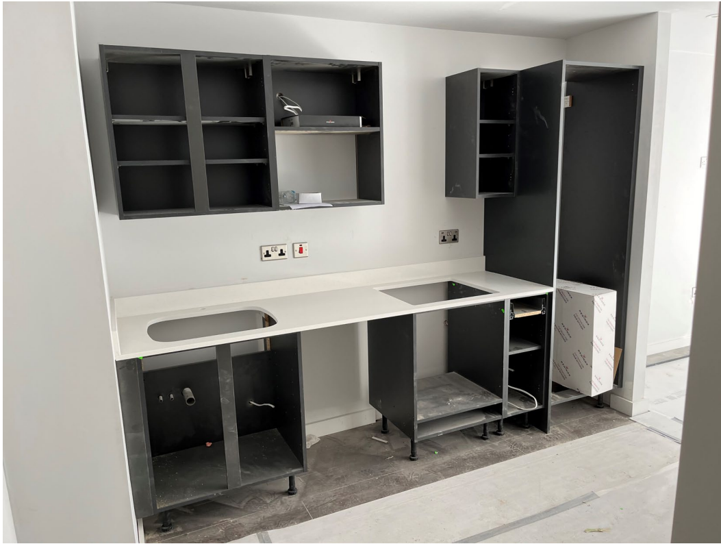
Installation of kitchen units and worktops ongoing
