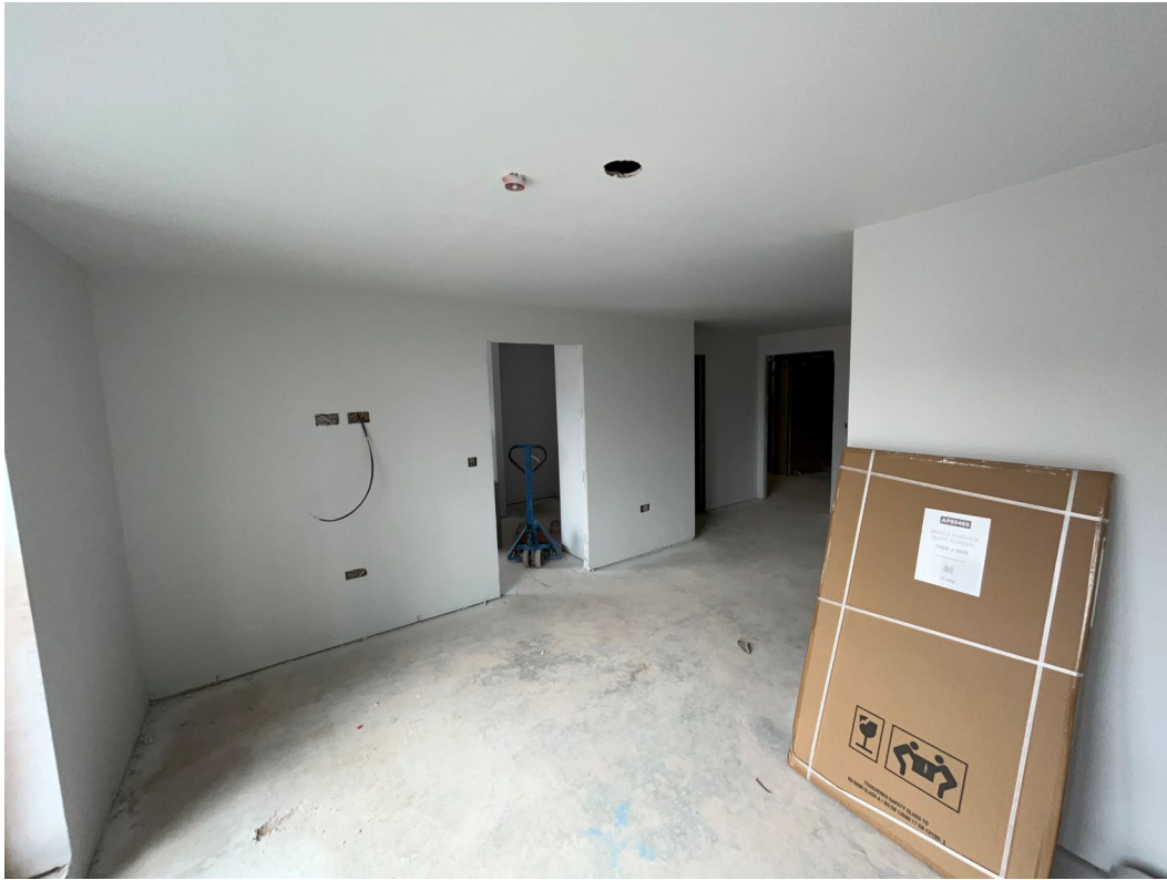
Internal finishes ongoing
