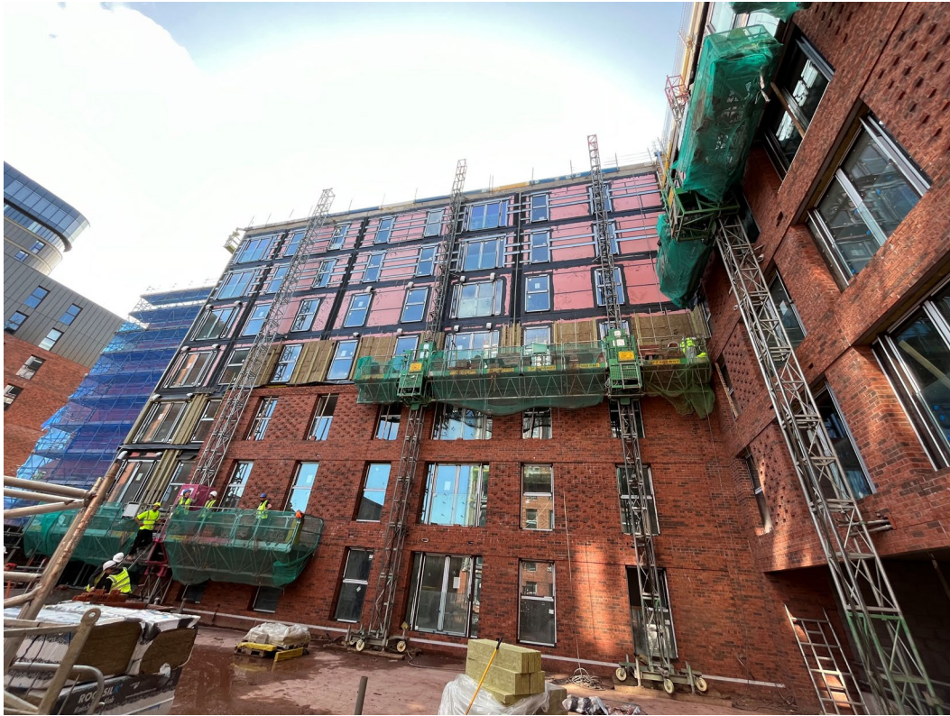
Block D Section B – Mast climbers
