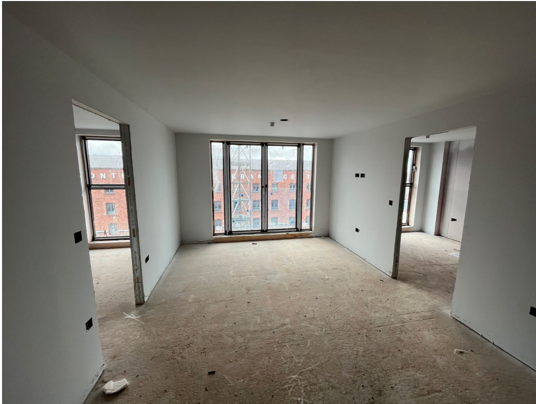
Walls and ceiling mistcoat application
