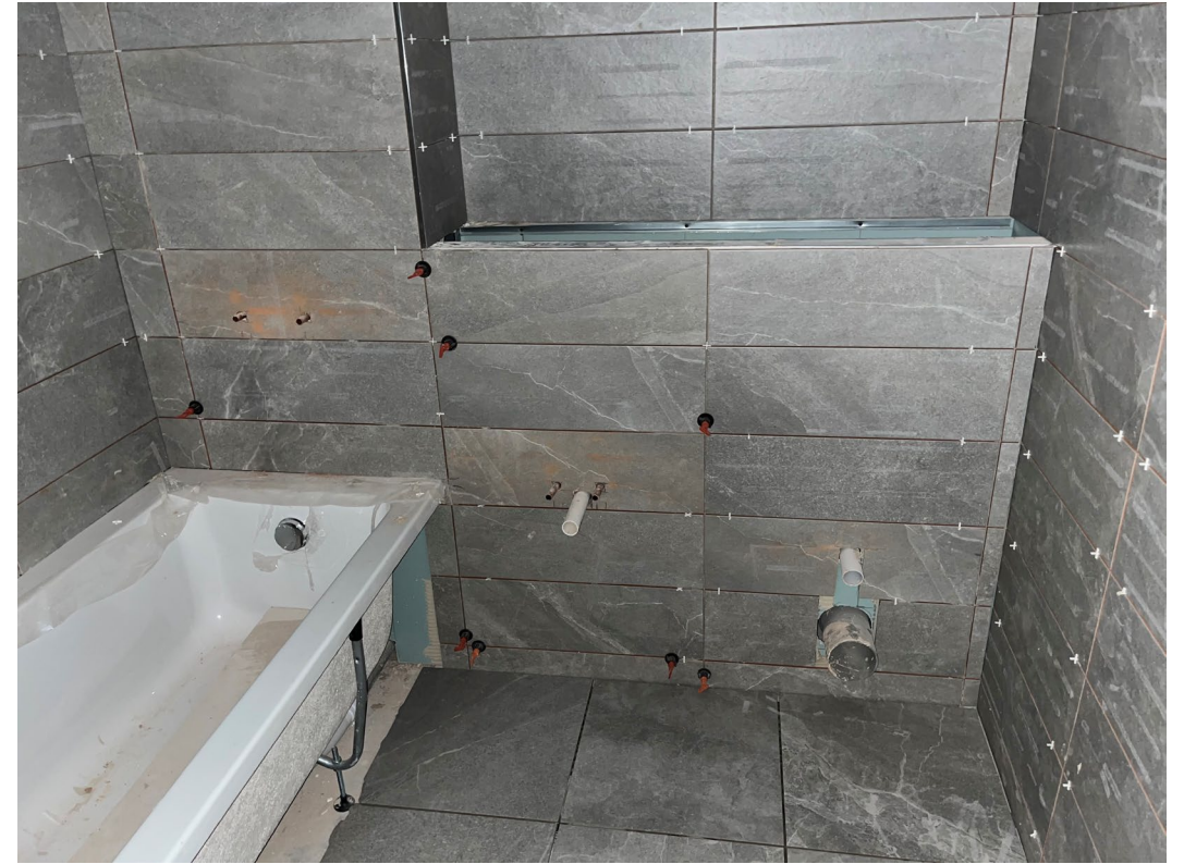
Wall and floor tile installation ongoing
