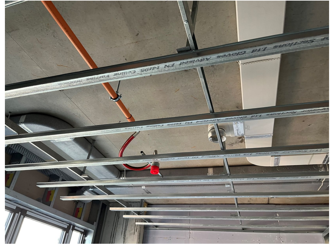
Metal ceiling grid installation ongoing
