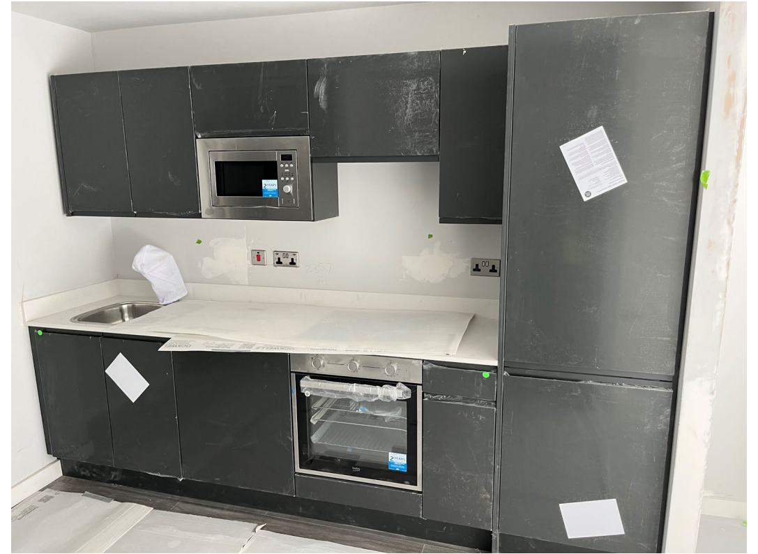
Installation of kitchen units and appliances ongoing
