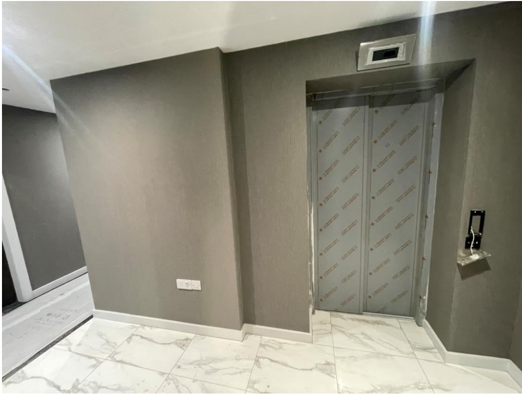
Wall coverings installed to lift lobby
