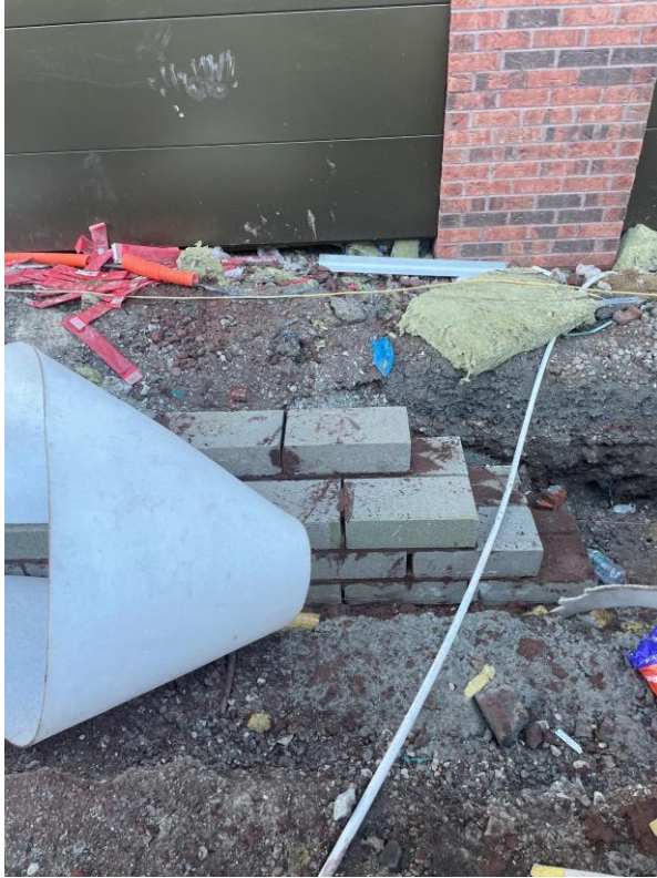
Blockwork installed to main entrance
