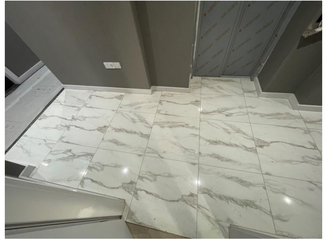
Tiled flooring to lift lobby
