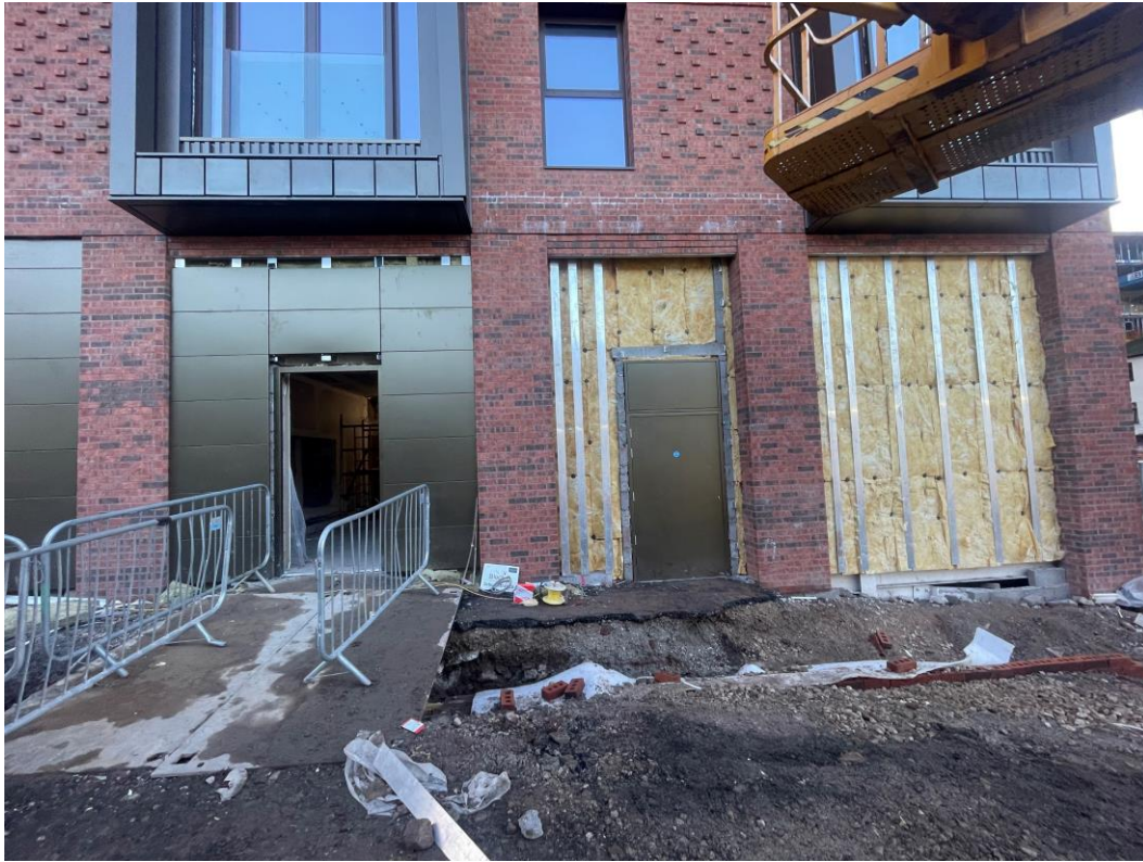
Cladding installation nearing completion
