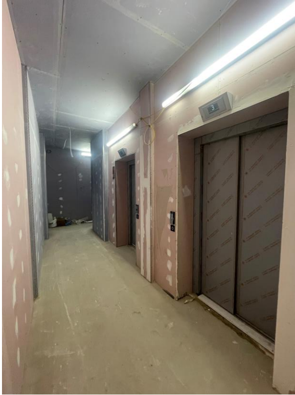
Boarding to lift lobby walls & ceilings
