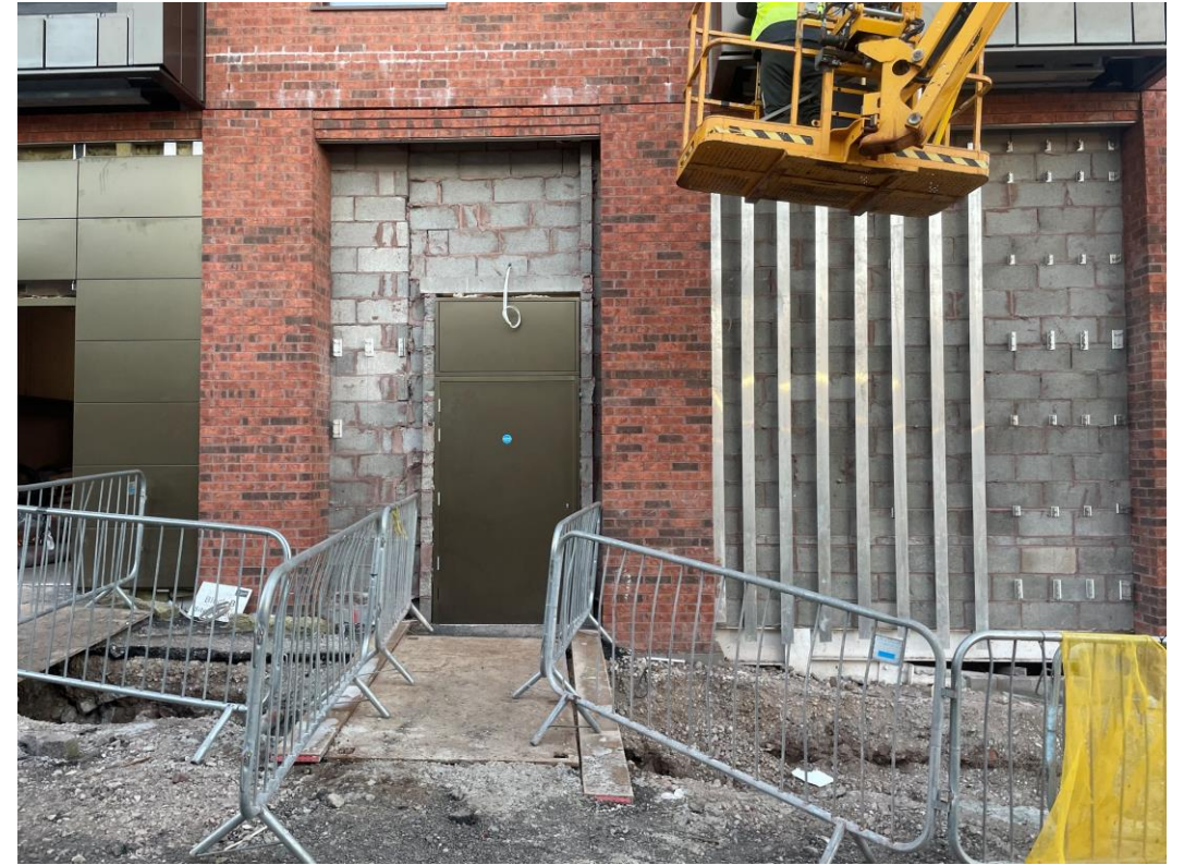
Cladding installation nearing completion
