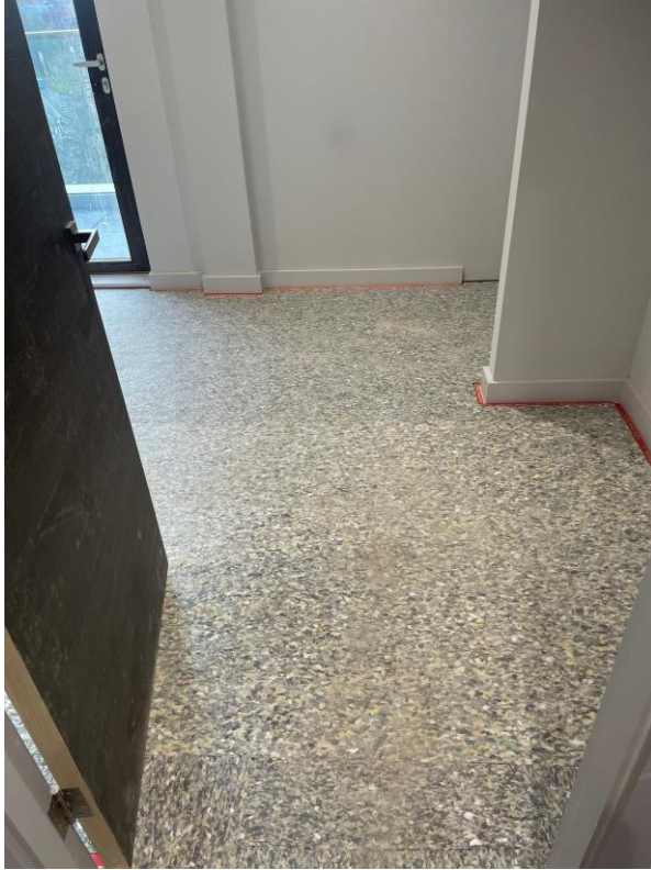
Underlay installed to bedroom in preparation for laying of carpets
