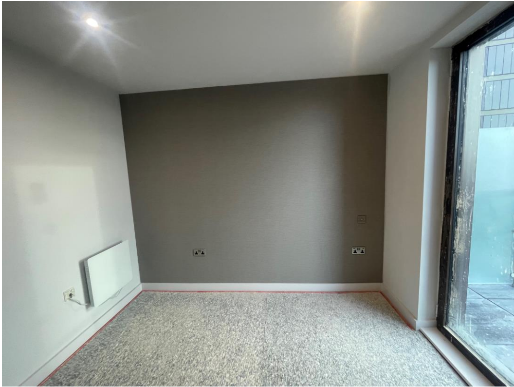
Wall coverings installed to bedroom
