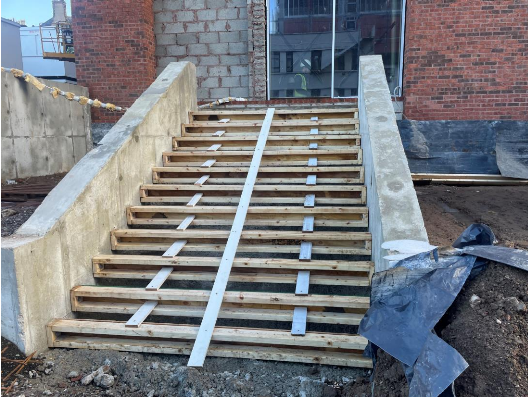
Formwork in place for casting of steps
