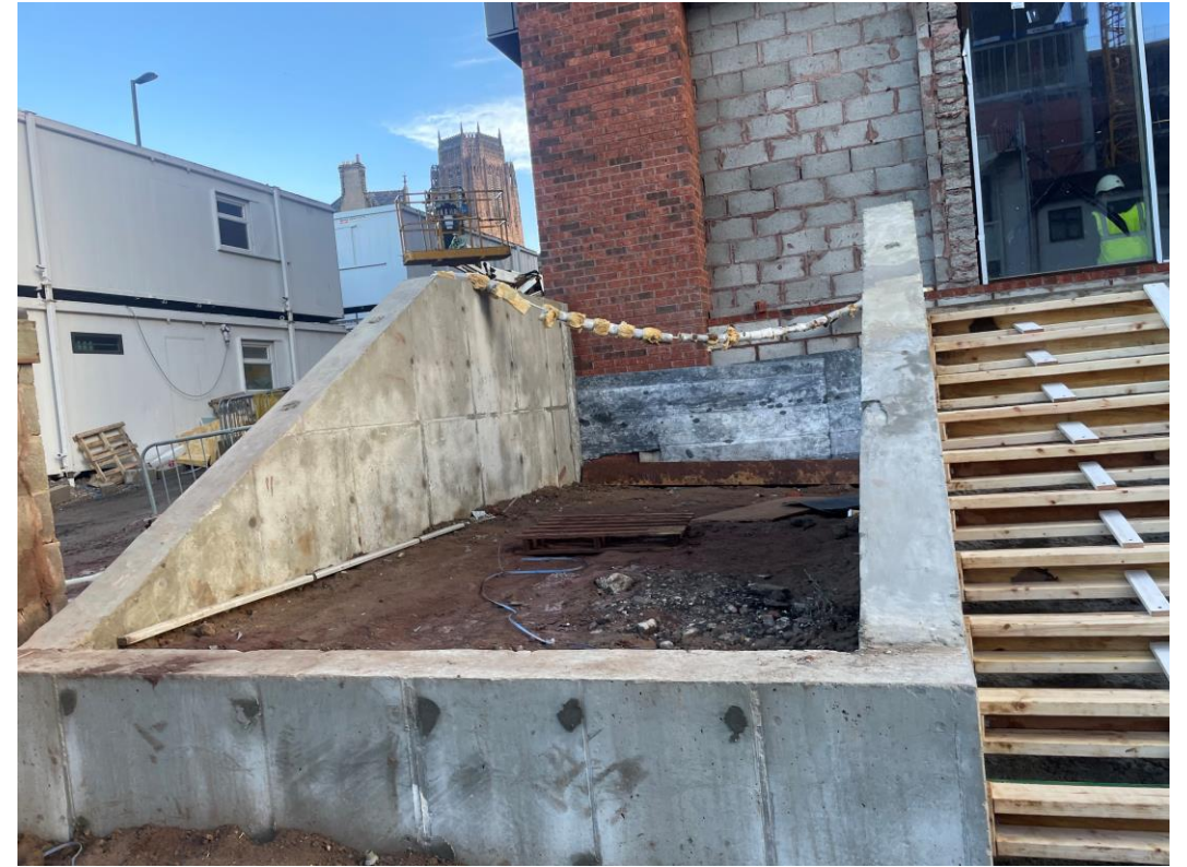
Retaining wall formed
