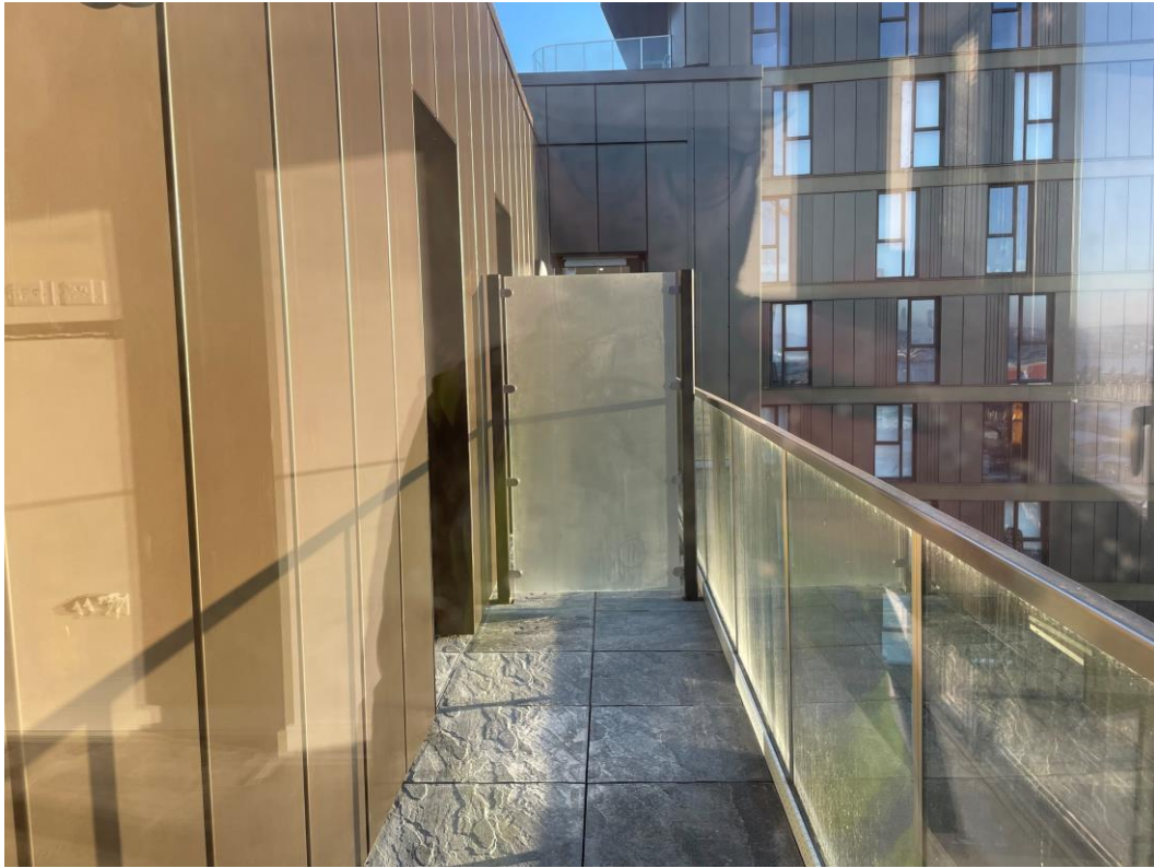
Balcony dividers installed
