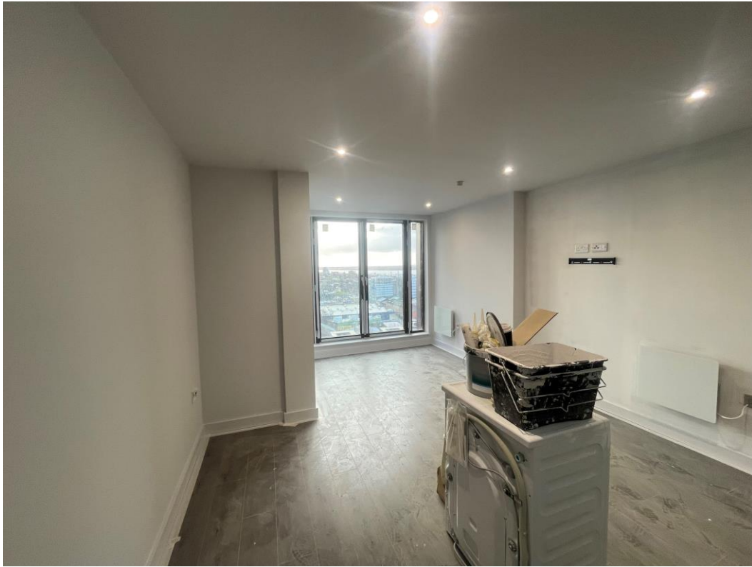
Decoration works complete to level 11 apartments
