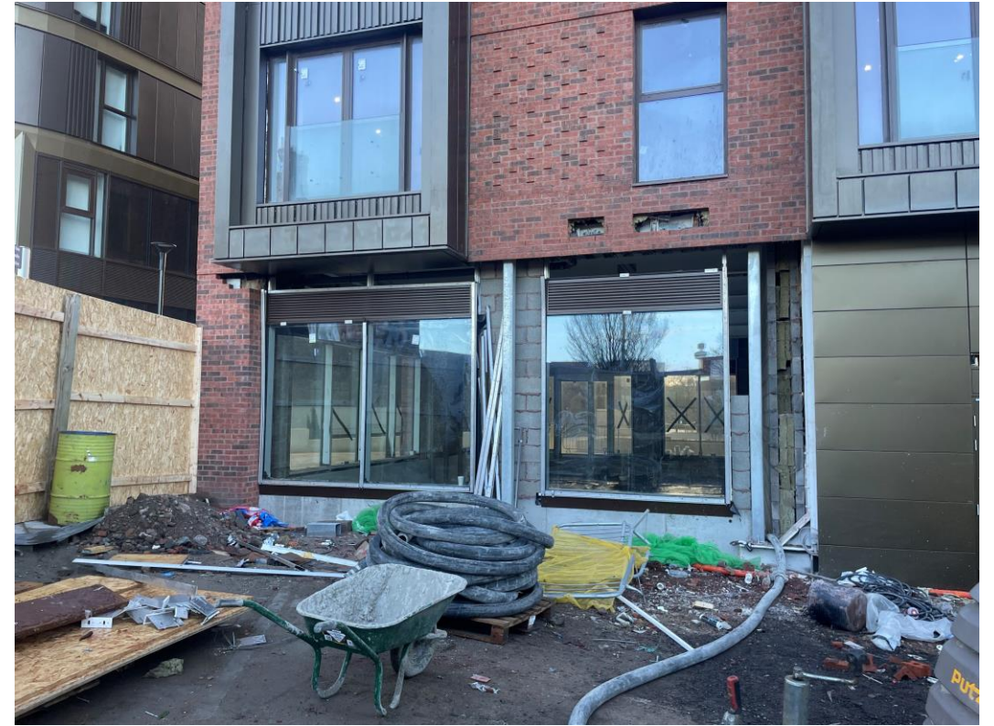
Curtain wall installation nearing completion
