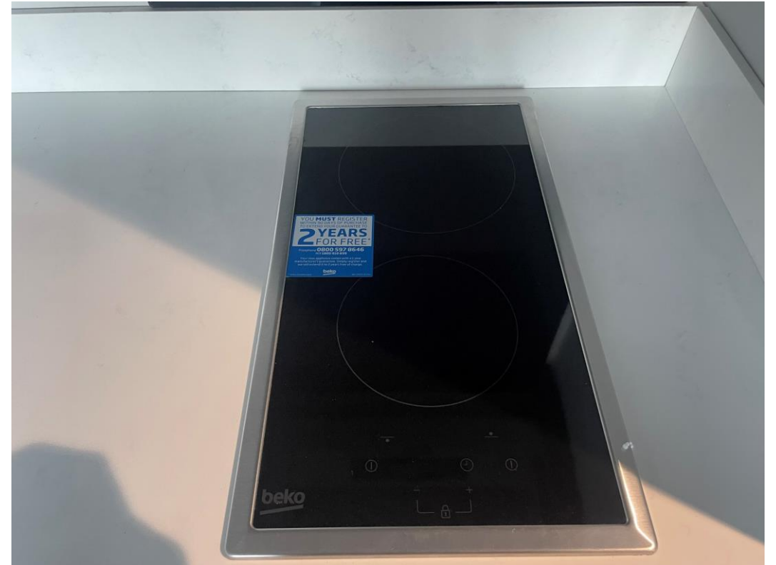
Electric hob installed
