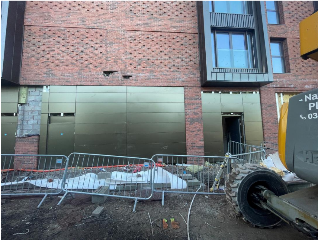
Cladding installation nearing completion
