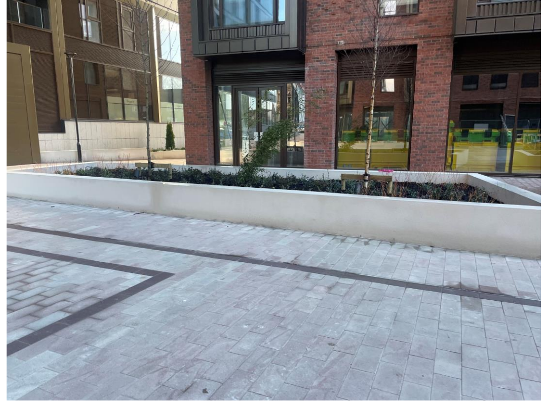
Planter construction complete
