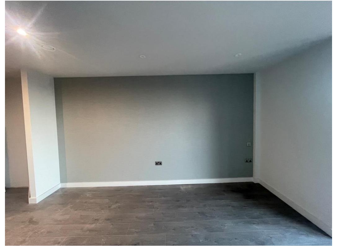
Wall coverings installed to lounge
