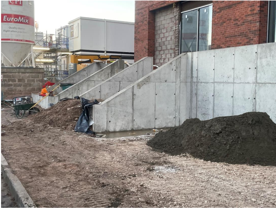
Retaining wall formed
