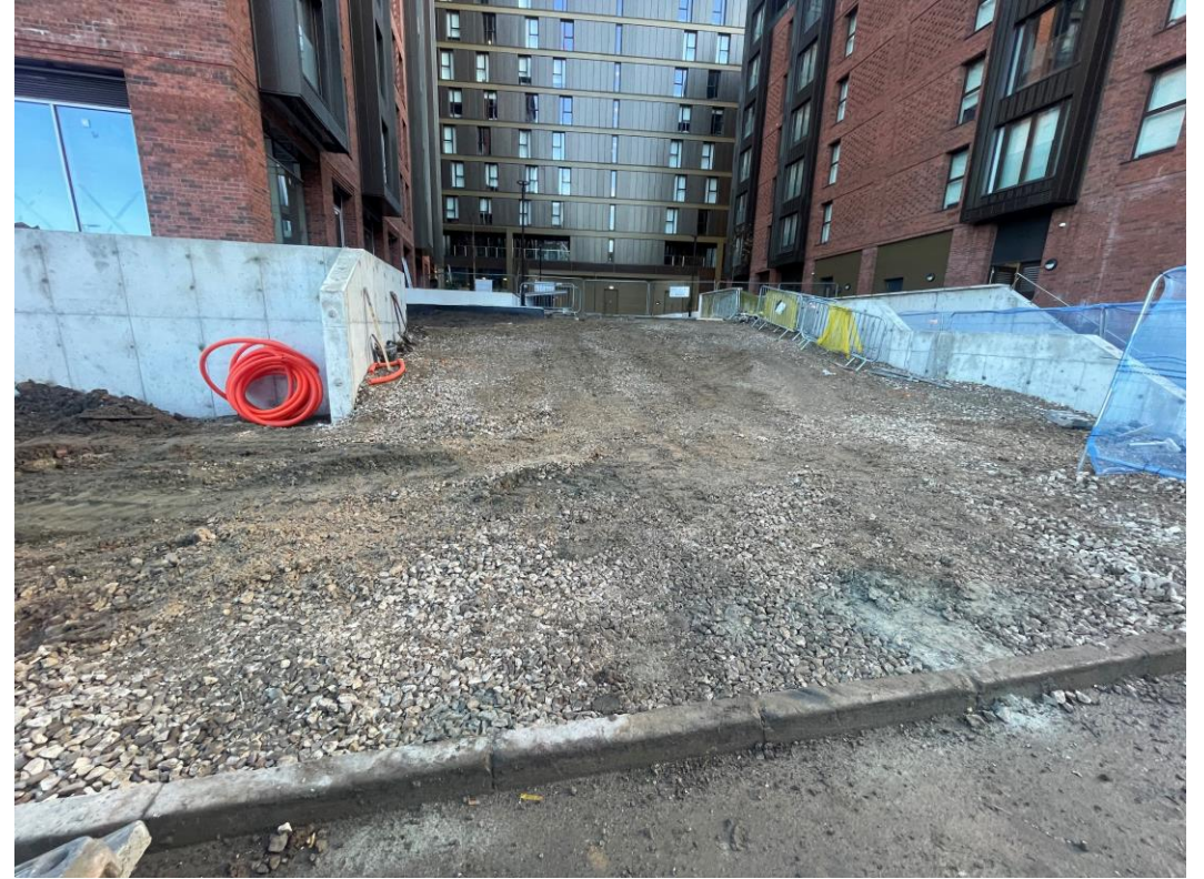
Formation for podium access ongoing
