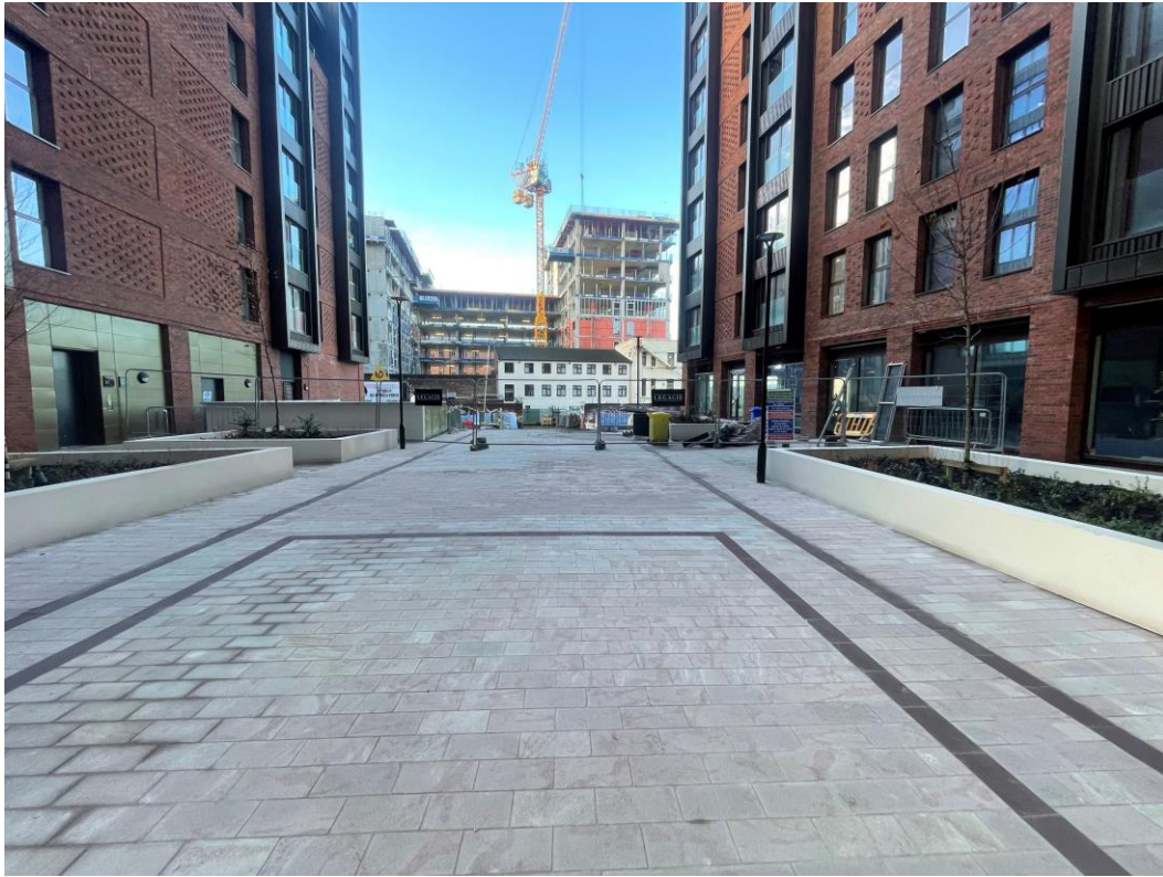
Paving flags installed
