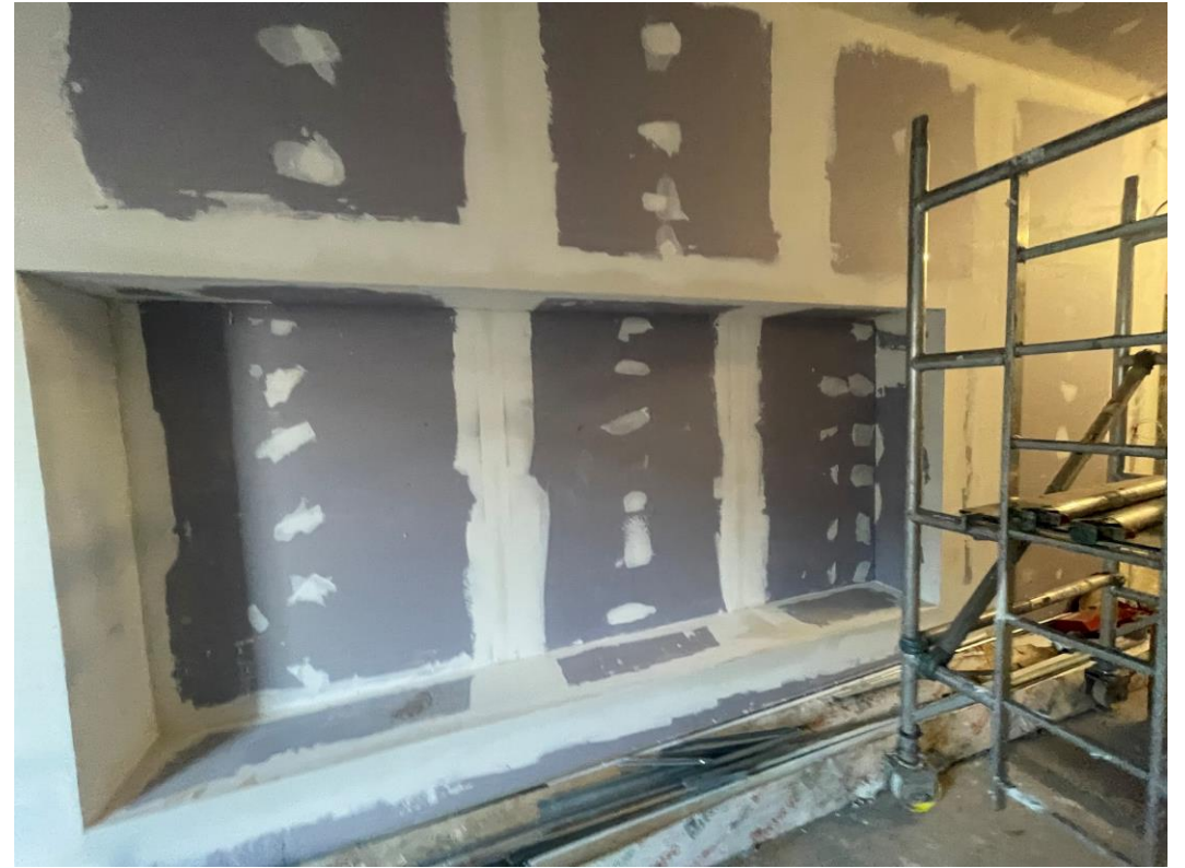
Tape & jointing ongoing
