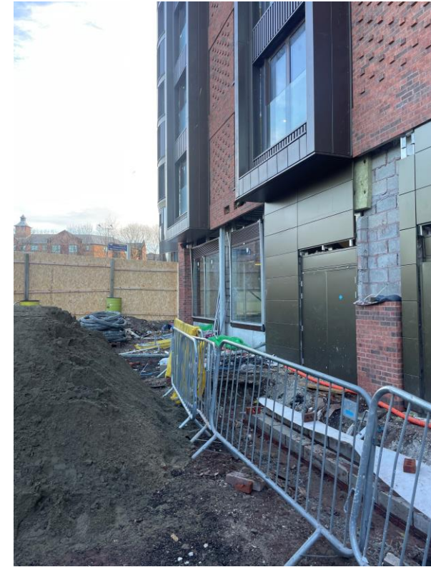
Cladding installation nearing completion
