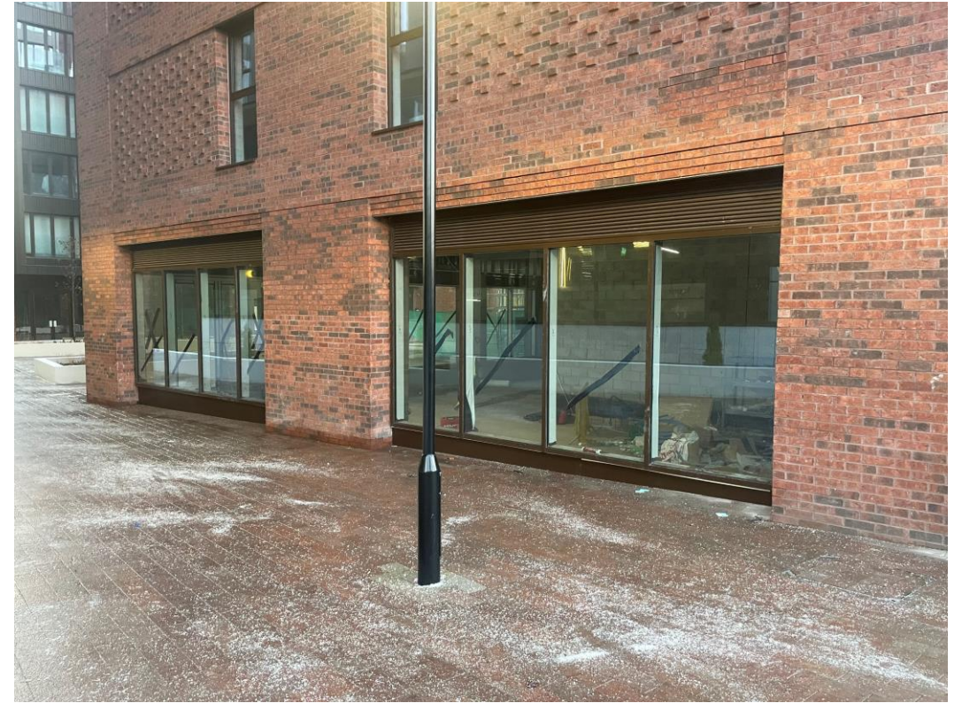
Block B - Curtain wall
