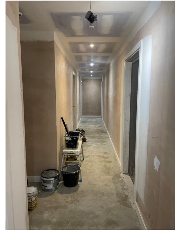
Screed applied to corridors
