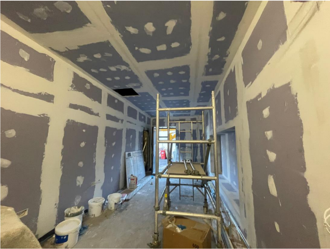
Tape & jointing ongoing
