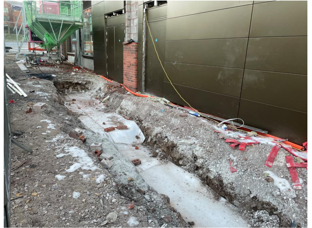
Footings poured for wall construction
