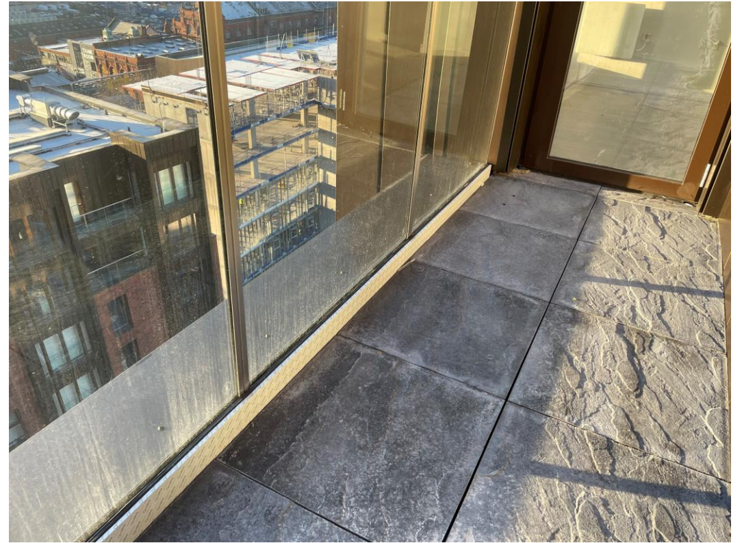
Balcony balustrades installed
