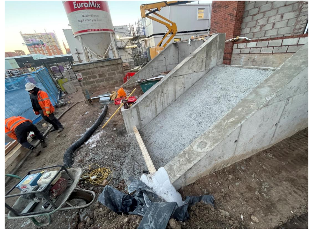
Retaining wall formed
