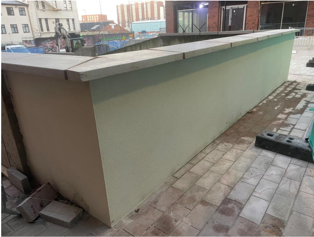
Copping stones installed
