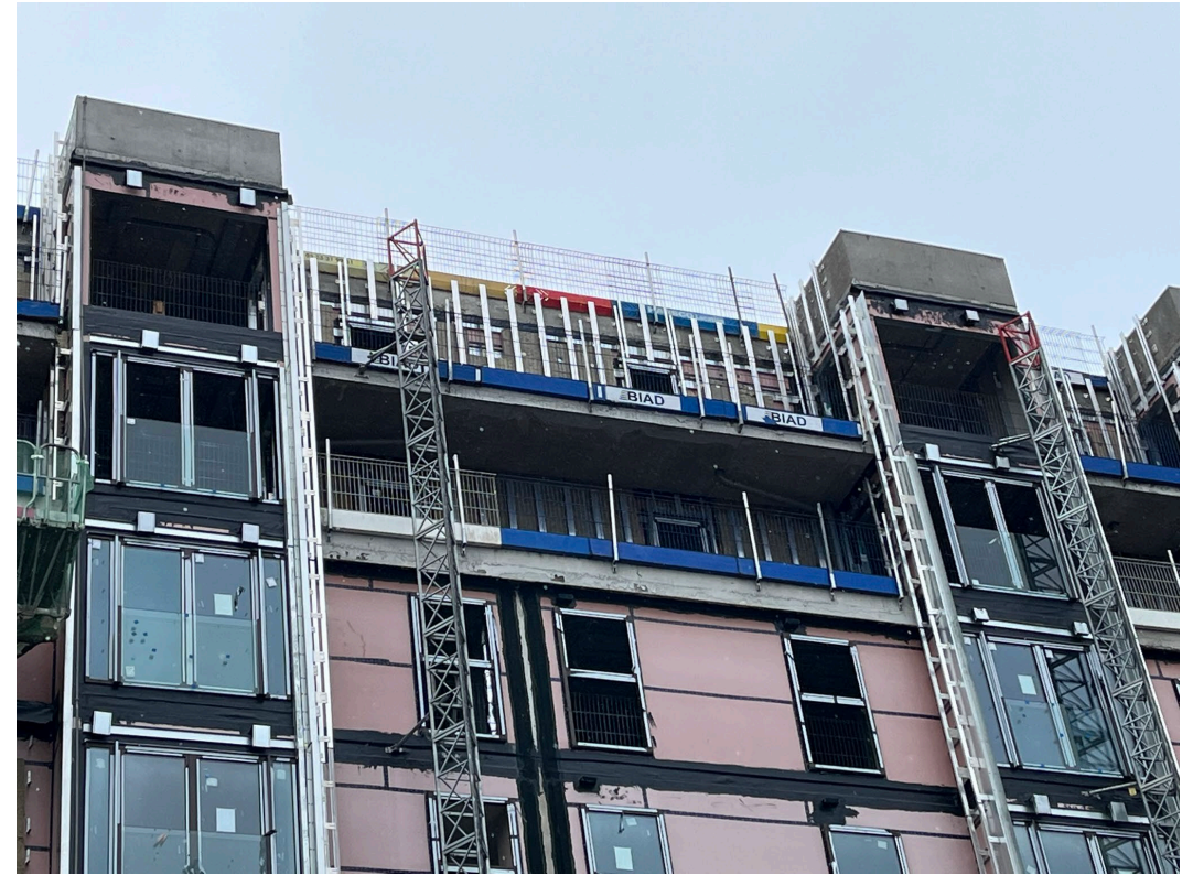
Block D Section B – Cladding bracket installation commenced
