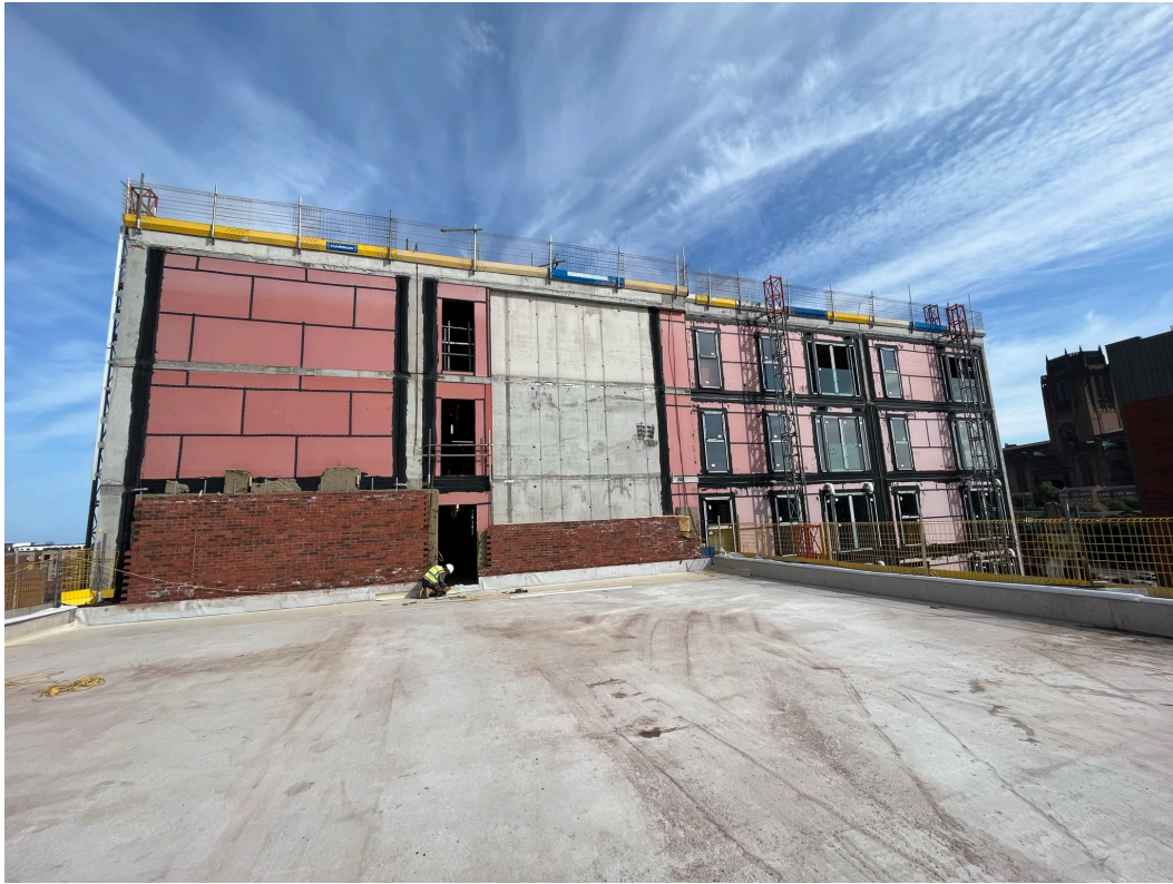
Block A – External brickwork and insulation installation
