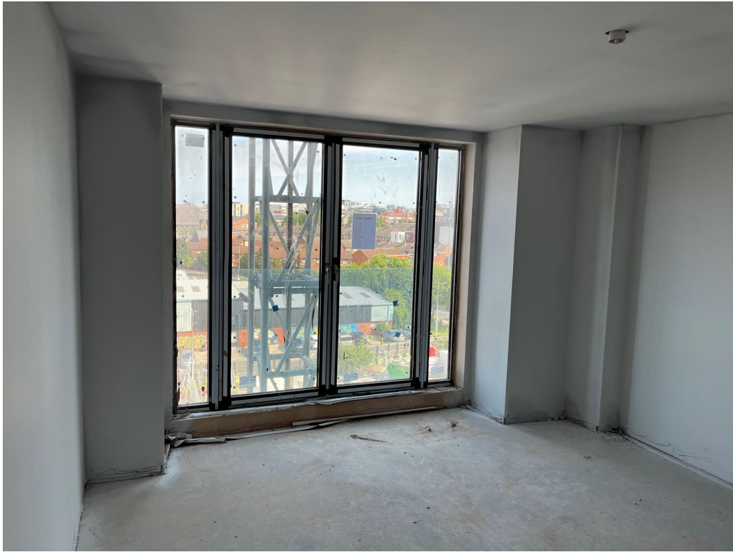
Internal finishes ongoing
