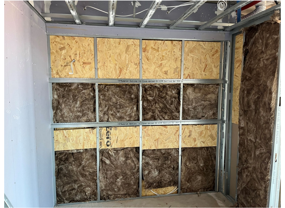
Insulation and pattress installation ongoing
