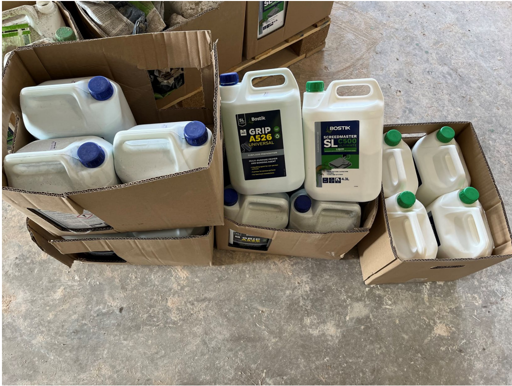
Screed binder onsite
