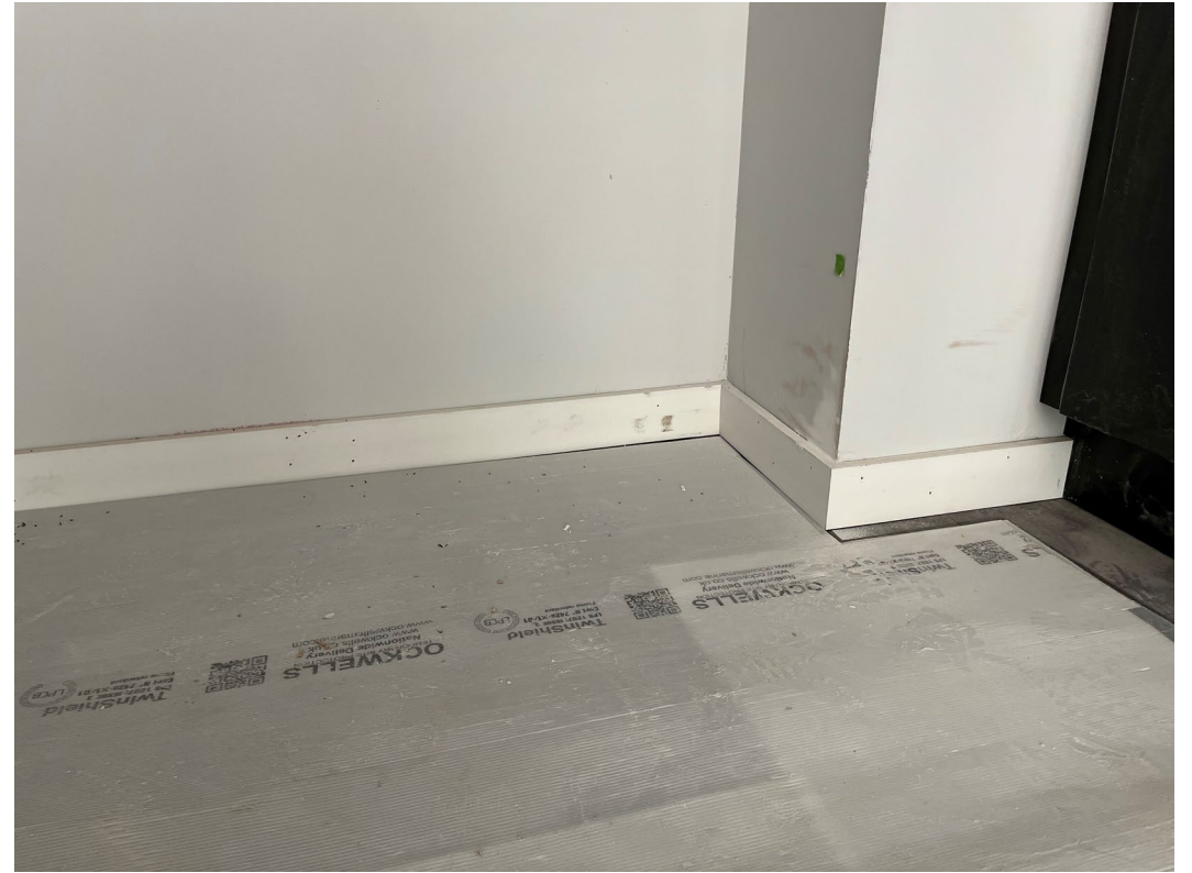
Timber skirting board installation ongoing
