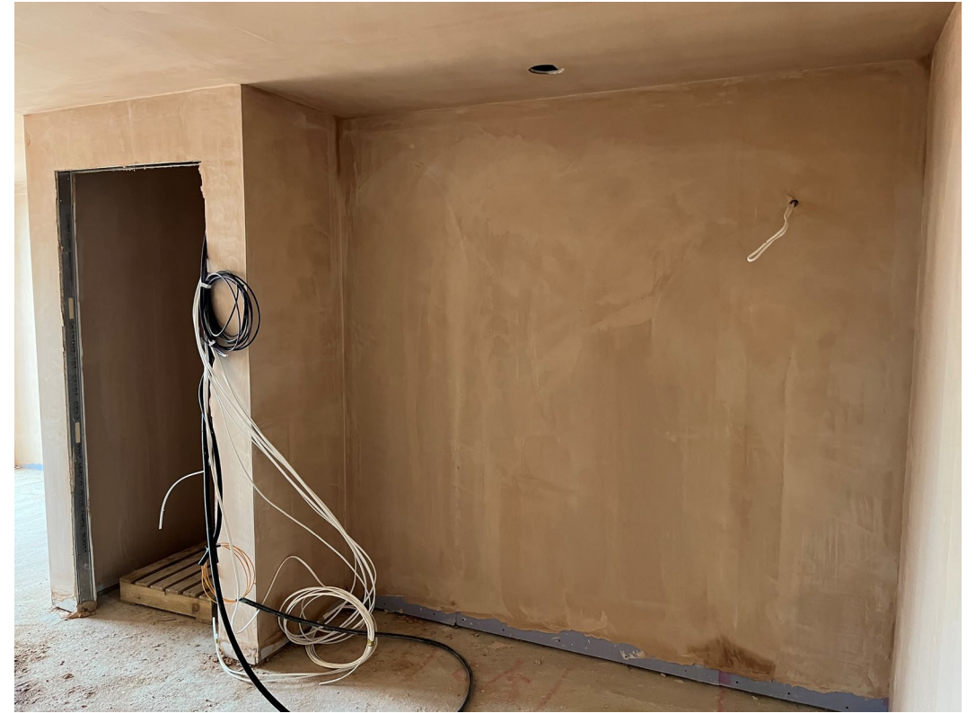
Plaster skim walls and ceiling application ongoing
