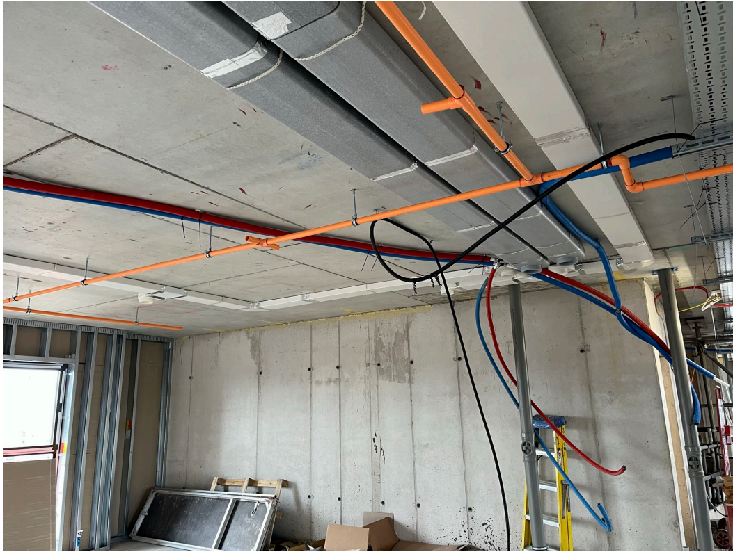
1 st fix mechanical ductwork installation ongoing
