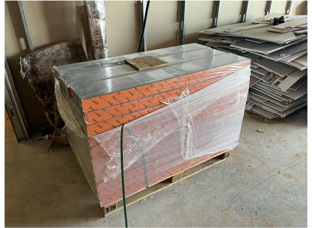
Laminate flooring onsite
