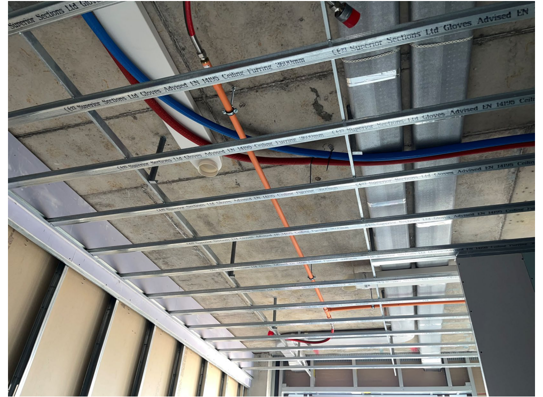
Metal ceiling grid installation ongoing
