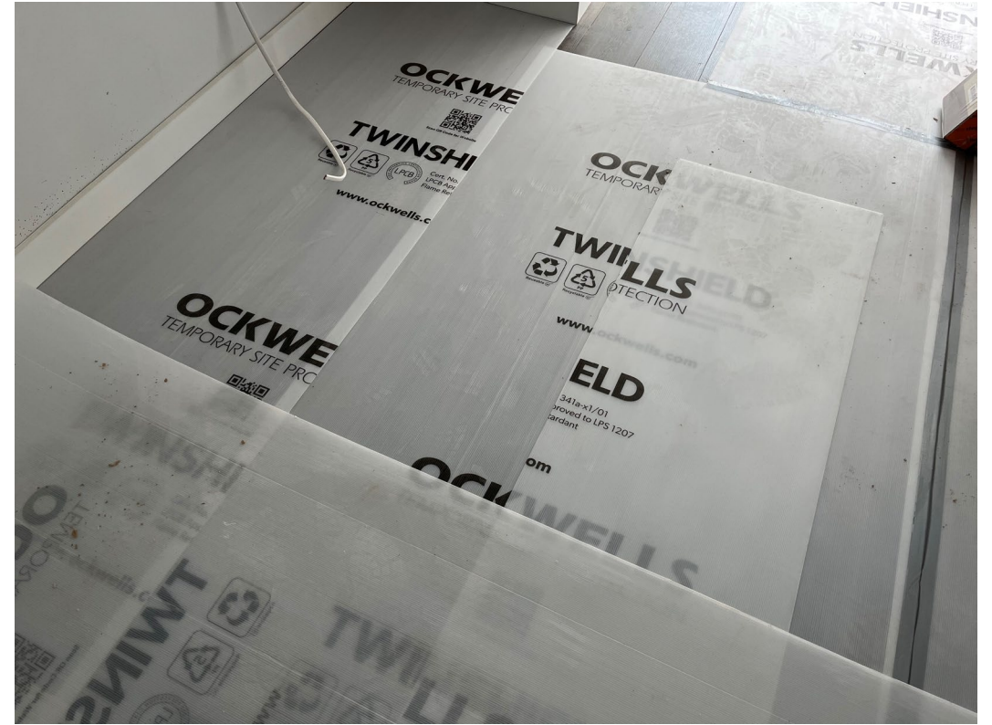
Laminate flooring installation and protection ongoing
