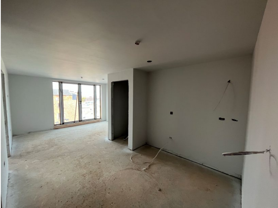
Walls and ceiling mistcoat application
