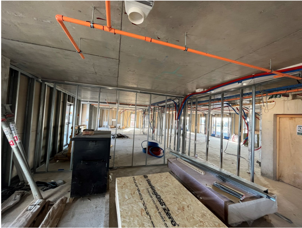
Erection of metal partition walls ongoing
