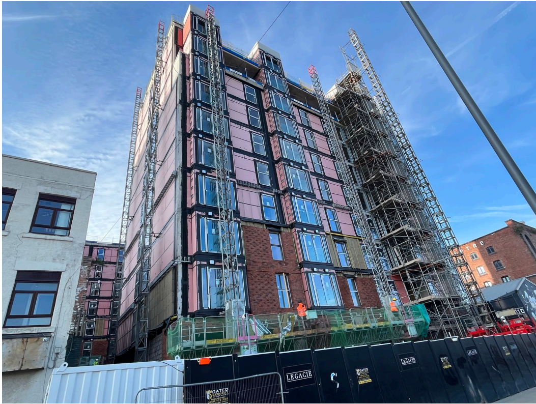
Block D Section A – Viewed from Greenland Street
