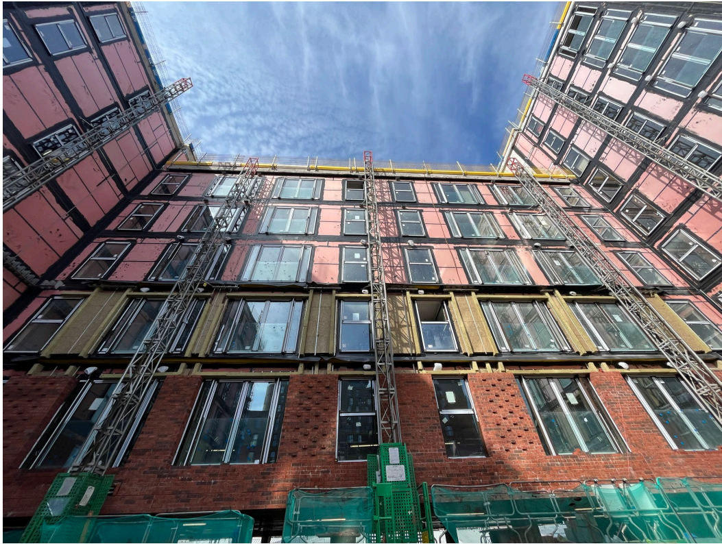
Block D Section C – Mast climbers
