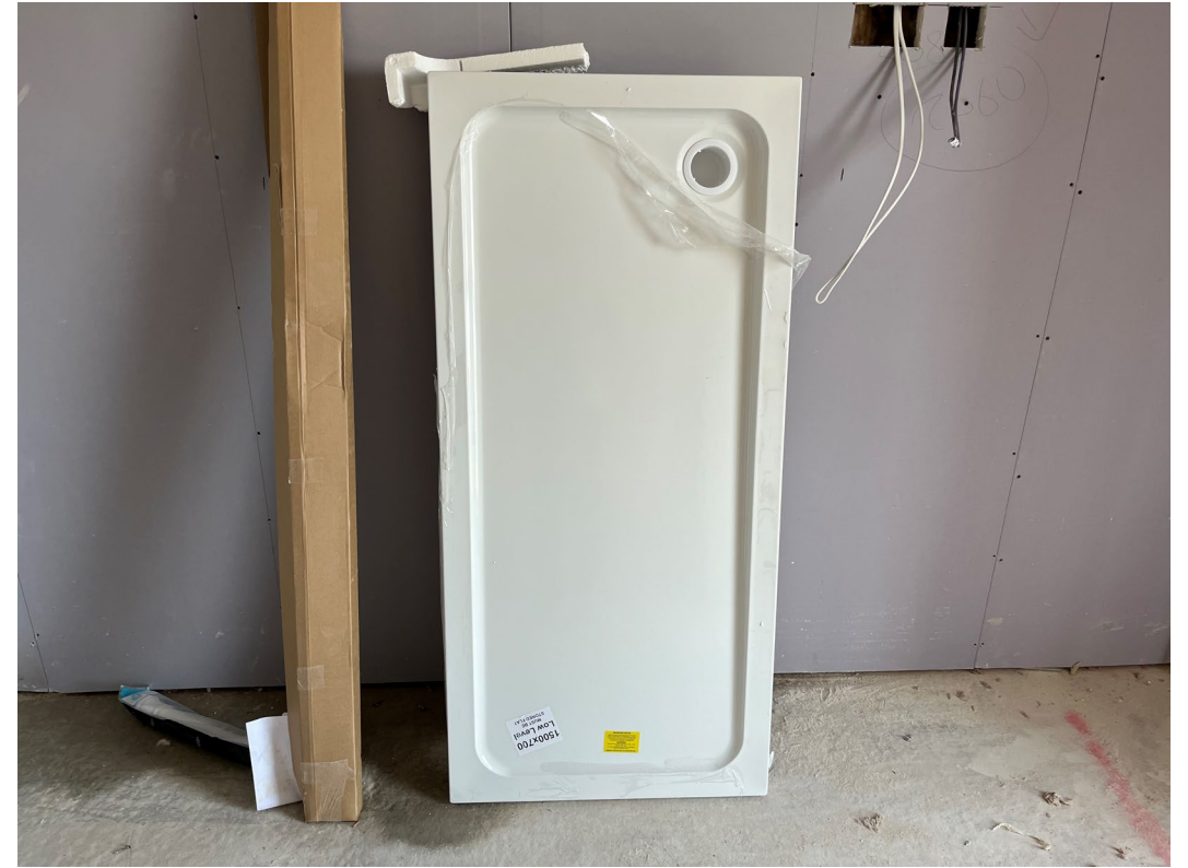
Shower tray onsite
