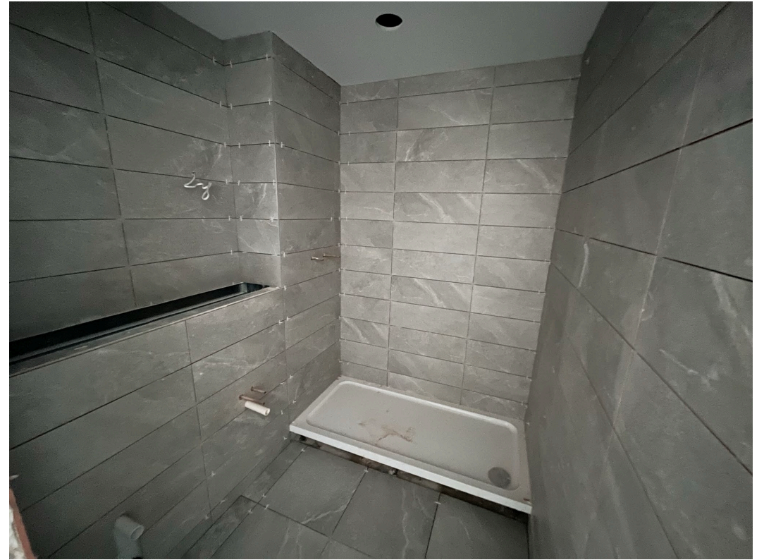
Wall tile installation ongoing
