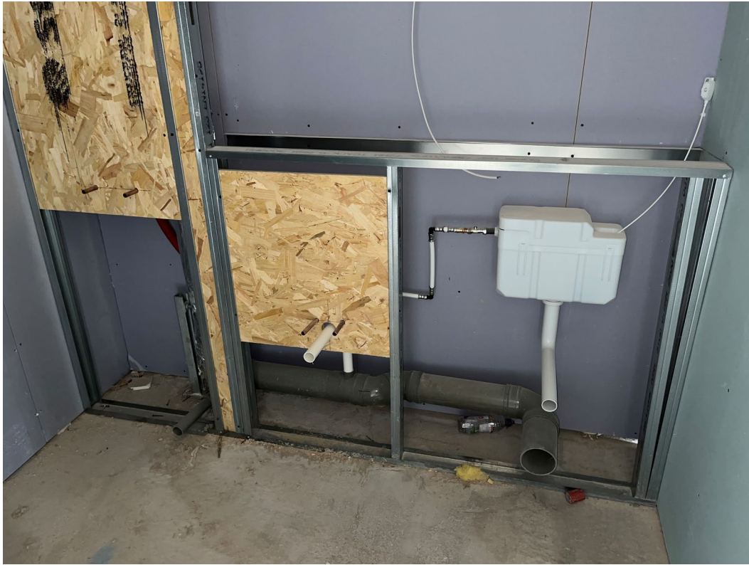
Pan installation and IPS ongoing
