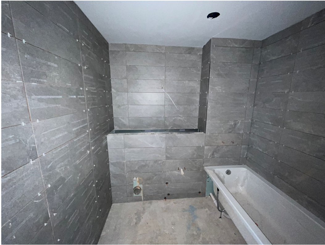
Wall tile installation ongoing
