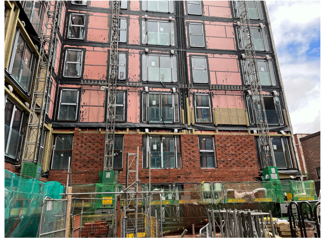
Block D Section A – Mast climbers
