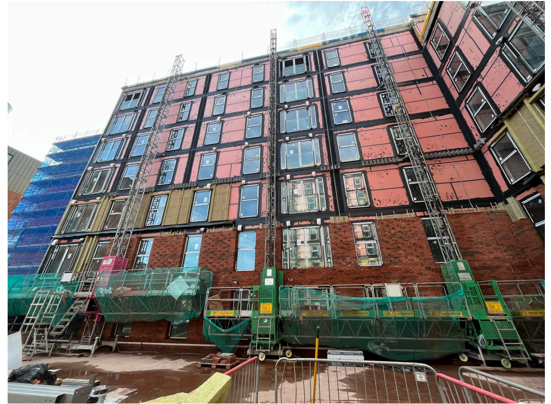
Block D Section B – SFS, weatherboarding & brickwork installation
