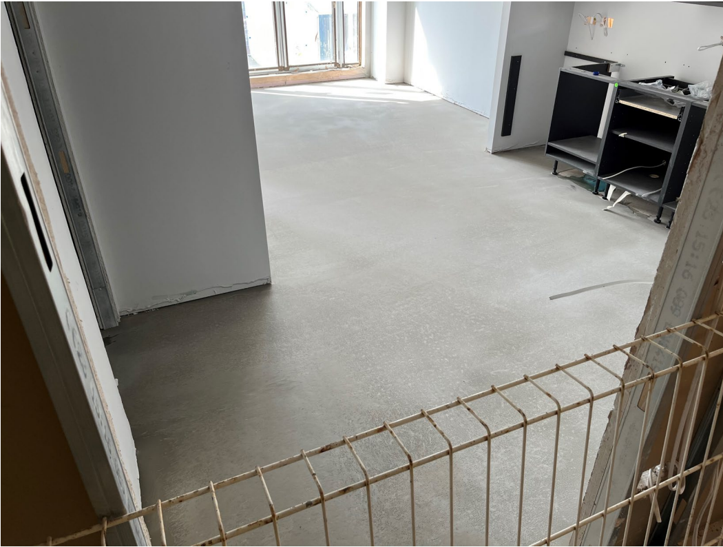
Self-levelling screed application ongoing
