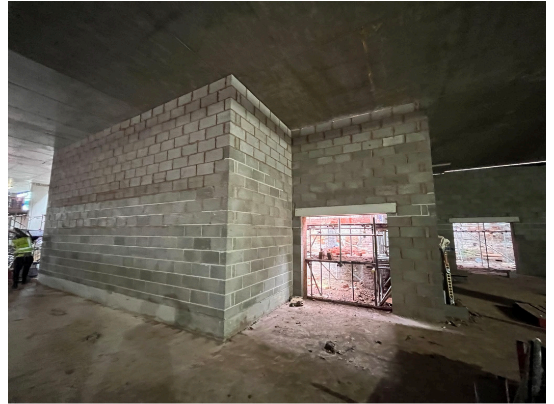
Internal blockwork ongoing
