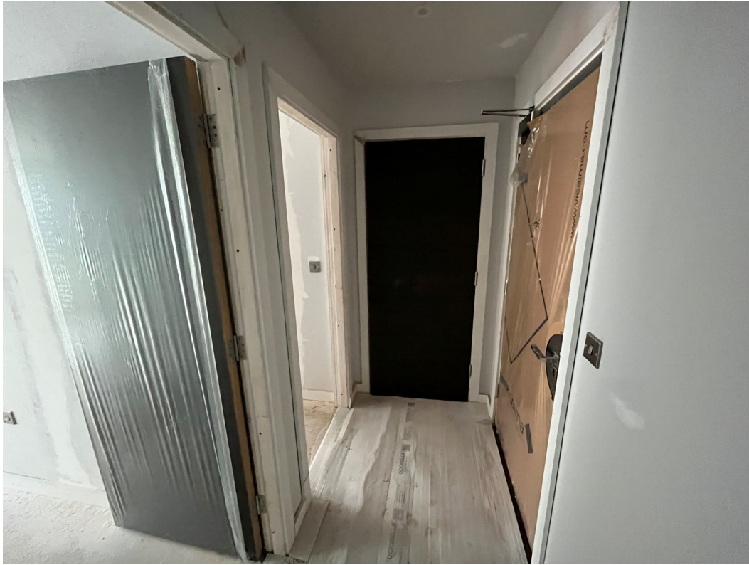
Internal joinery and doors installation ongoing
