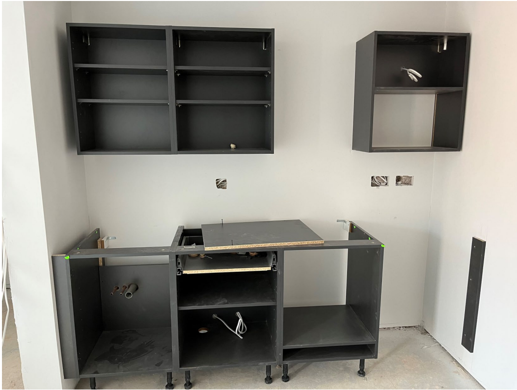
Installation of kitchen units ongoing
