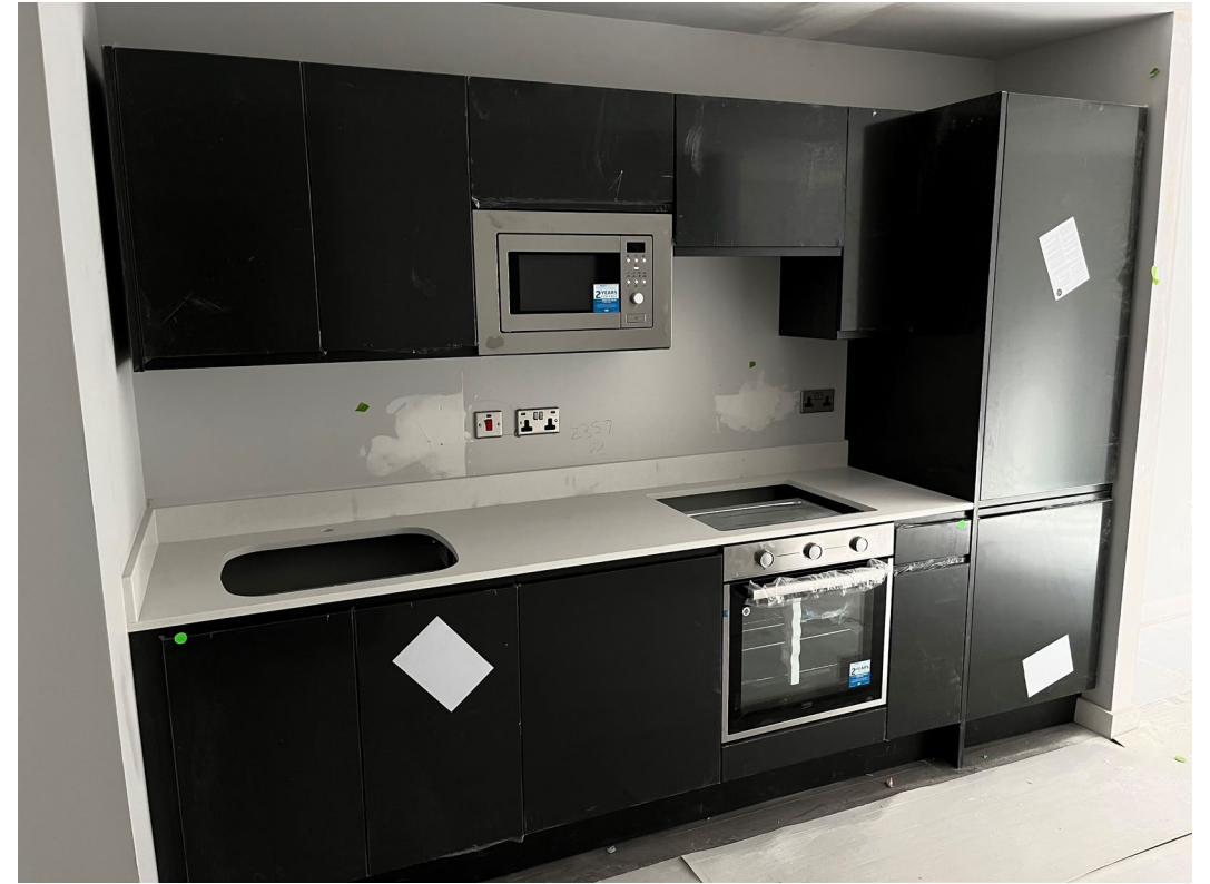
Installation of kitchen units and appliances ongoing
