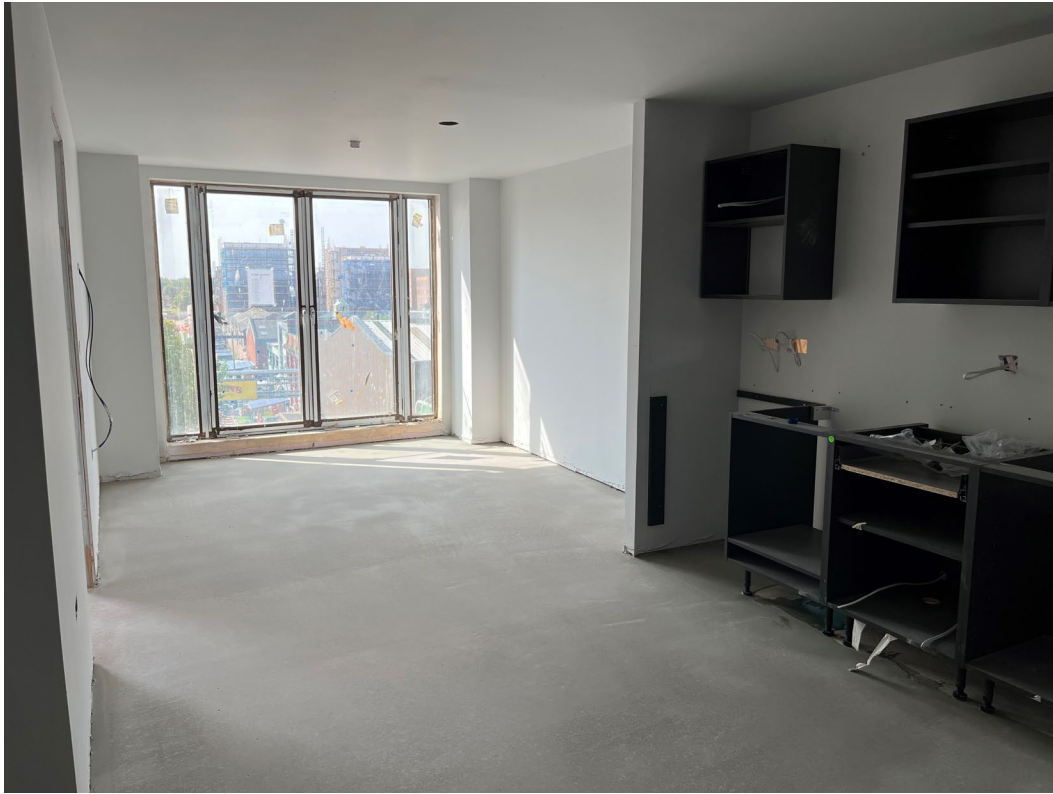
Internal finishes ongoing
