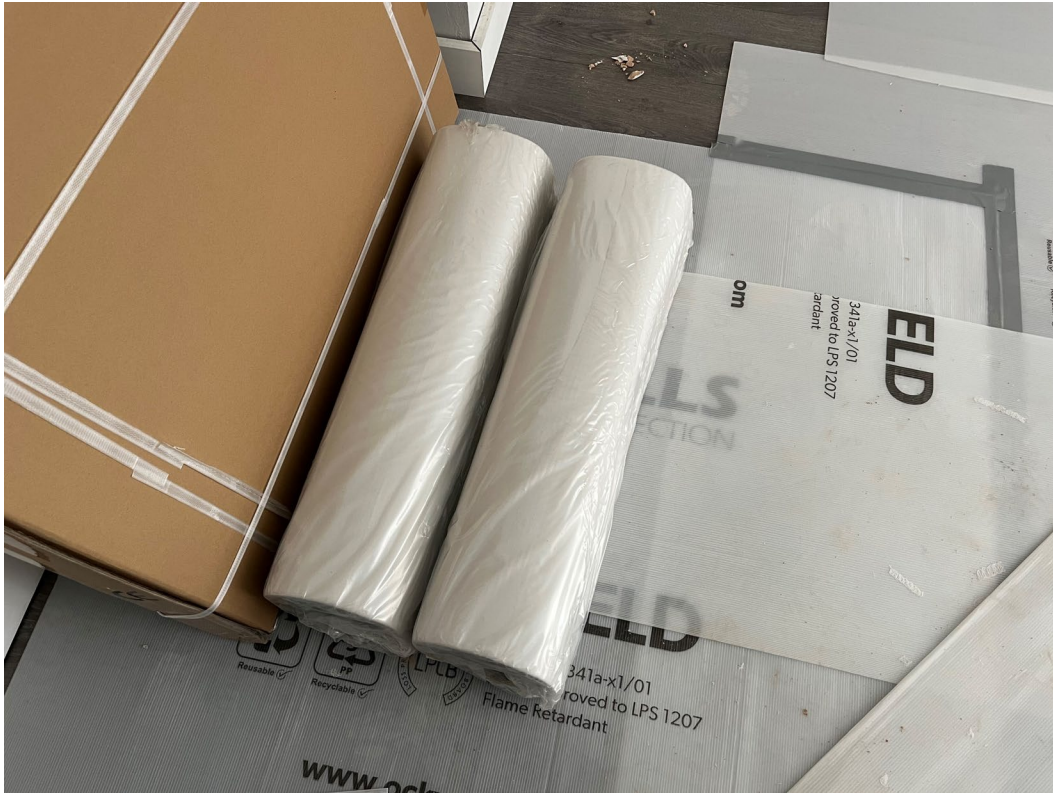
Sink pedestal onsite
