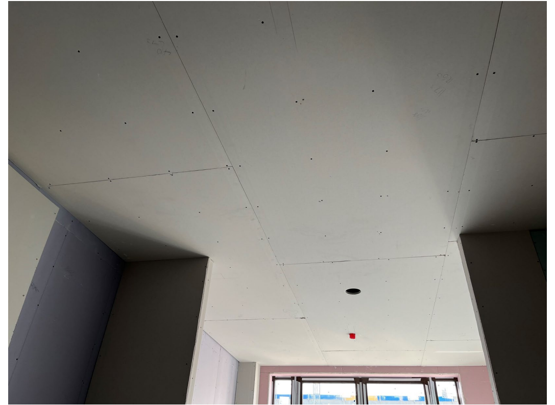
2 nd side boarding of ceilings ongoing
