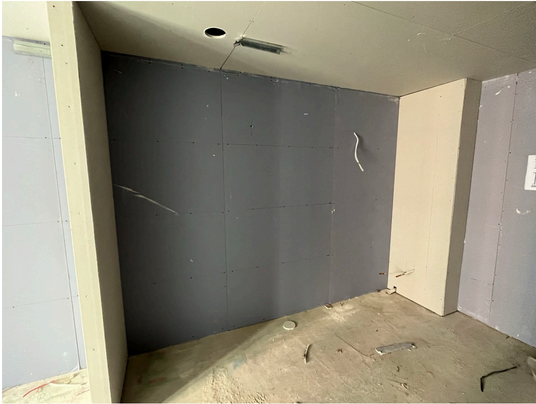
2 nd side boarding of walls ongoing
