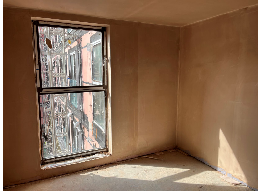
Plaster skim walls and ceiling application ongoing
