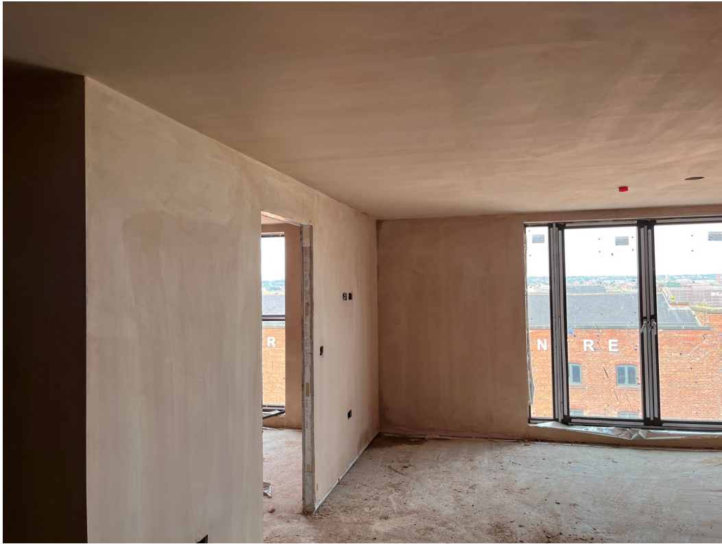
Plaster skim walls and ceiling application ongoing
