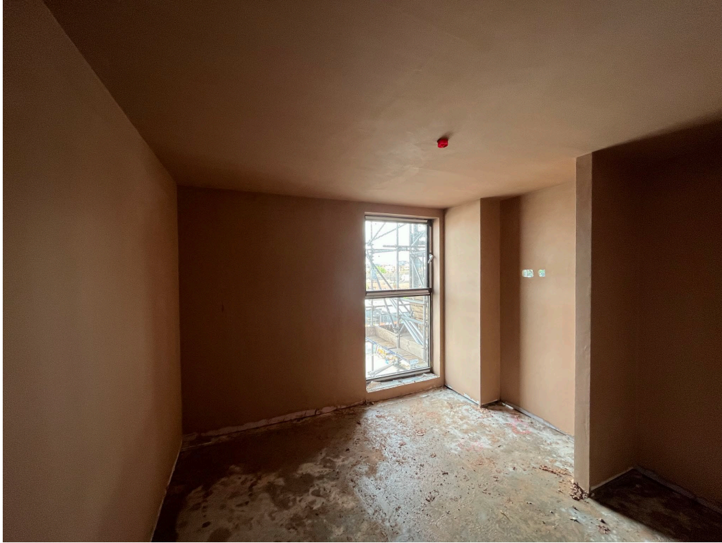
Plaster skim walls and ceiling application ongoing
