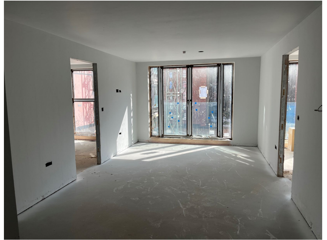
Internal finishes ongoing
