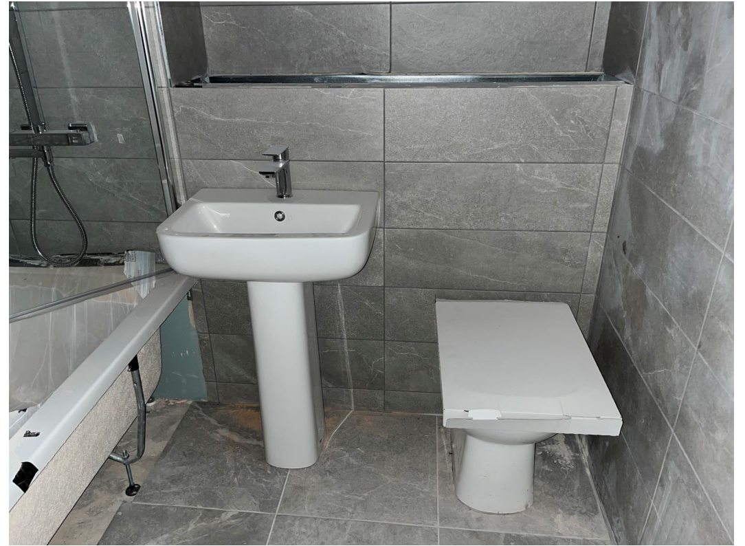
Sanitaryware installation ongoing
