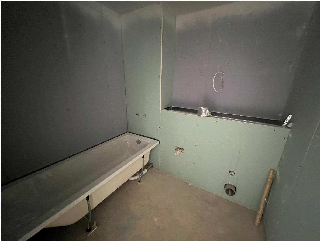
Sanitaryware installation ongoing
