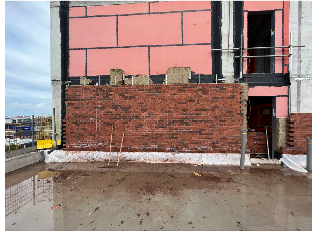
Block D – External brickwork and insulation installation
