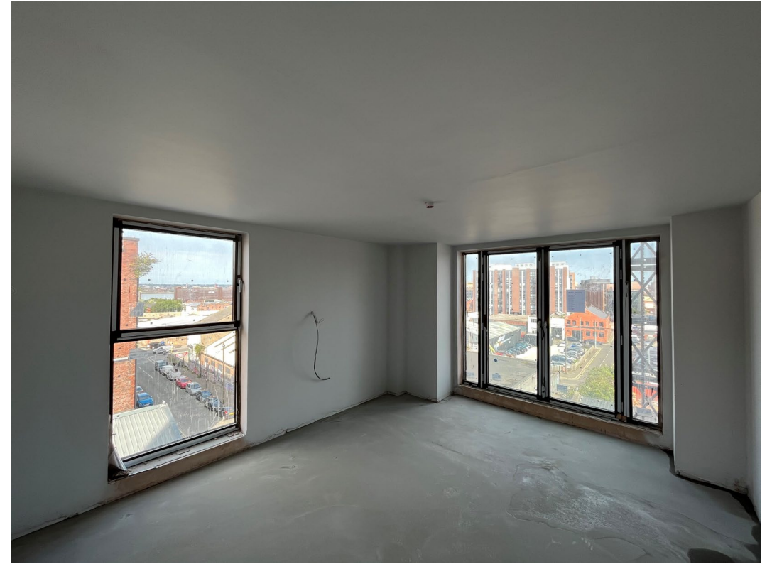
Internal finishes ongoing
