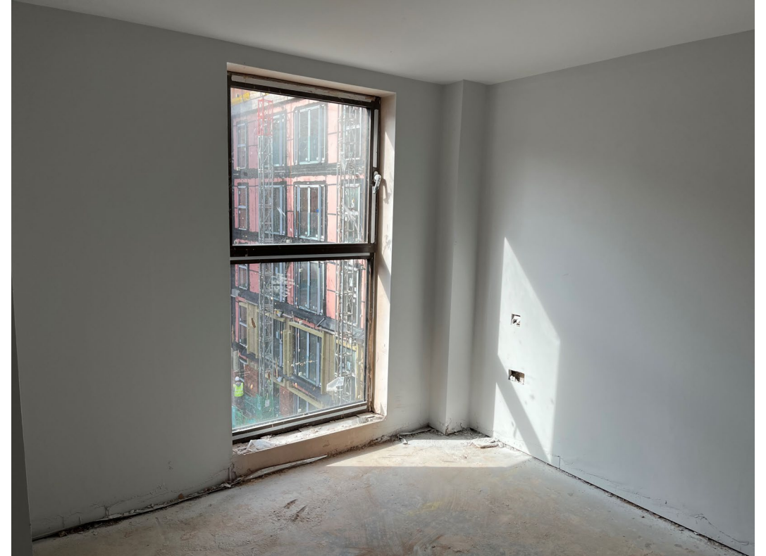
Walls and ceiling mistcoat application
