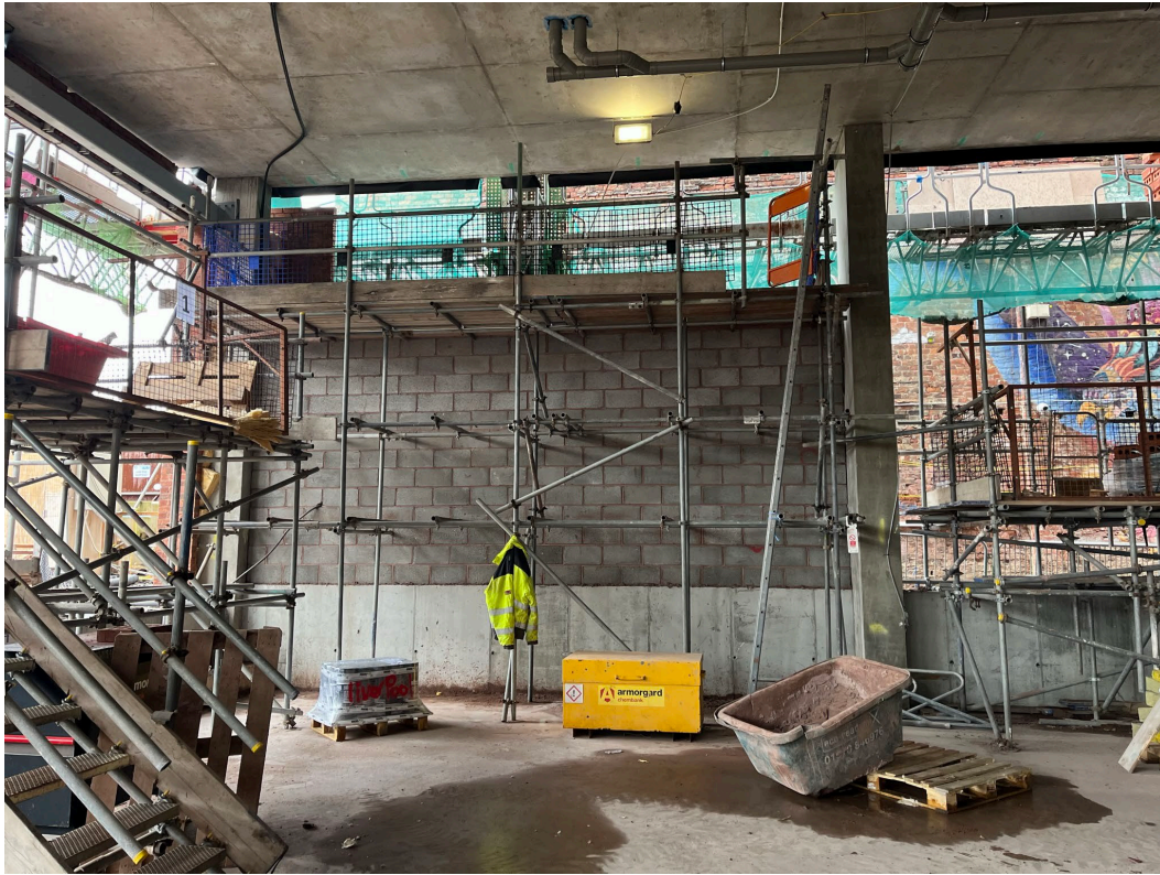
External blockwork ongoing
