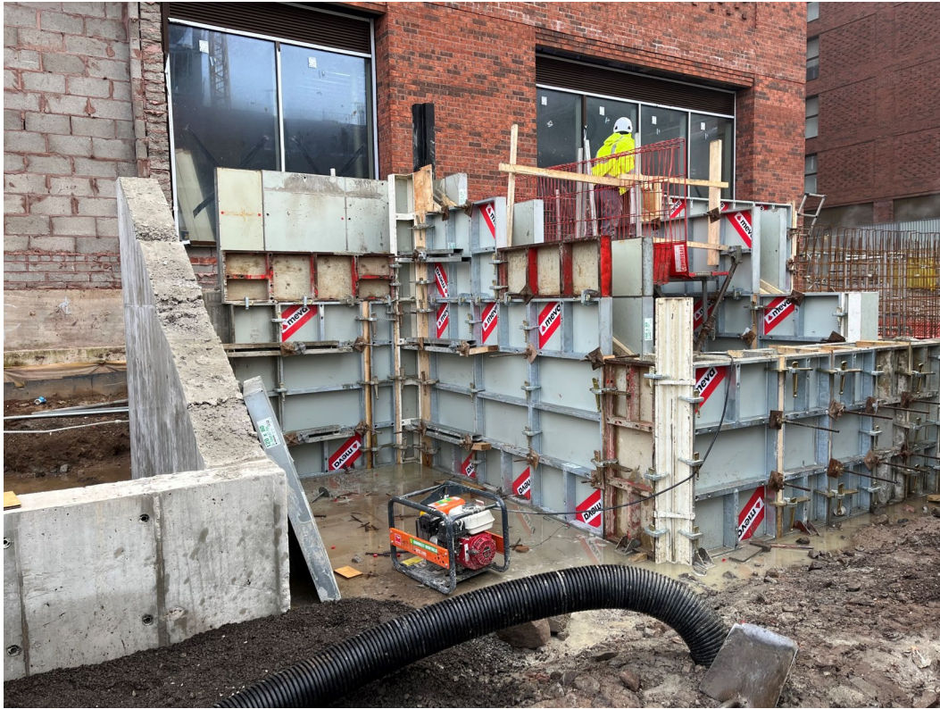
Formwork for retaining walls
