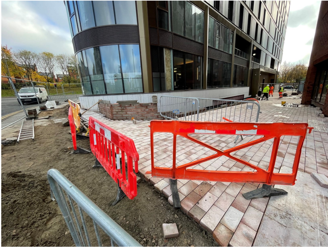
Paving works ongoing
