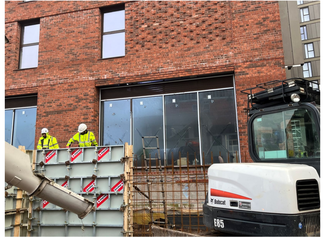
Curtain wall installation nearing completion
