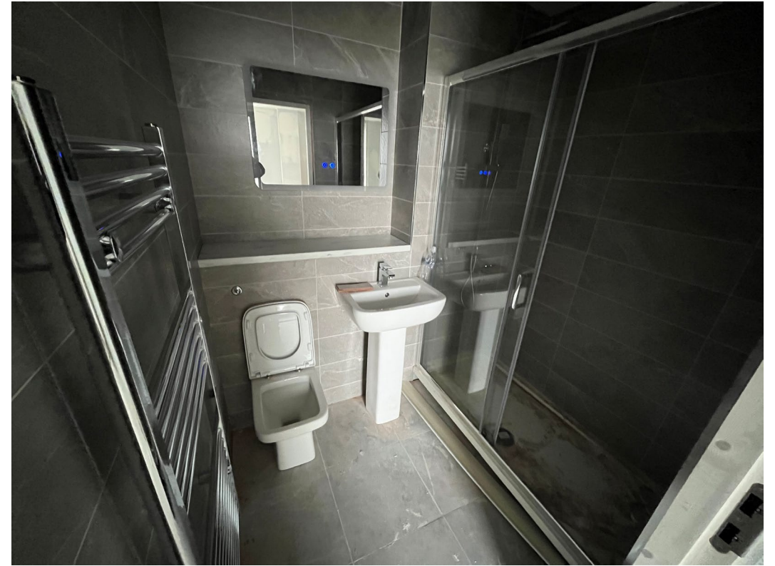
En-suite installation nearing completion
