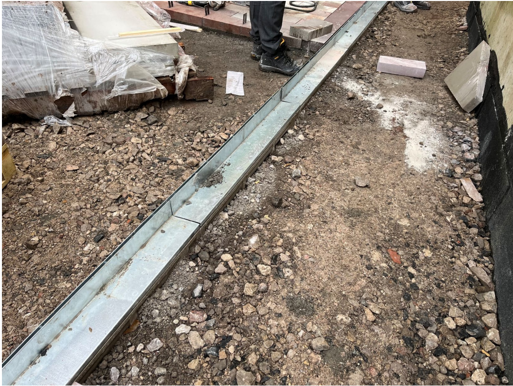
ACO Slimline Drains installed
