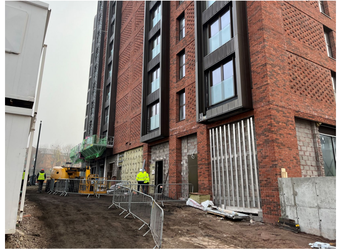
Brickwork façade nearing completion
