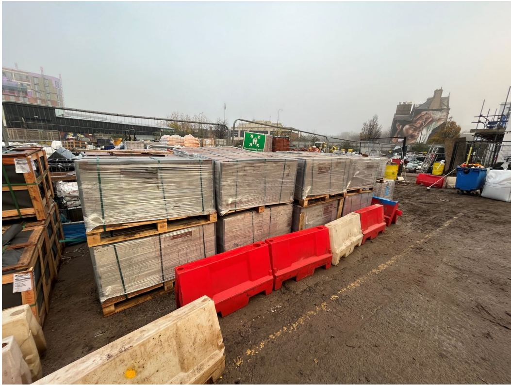
Paving on site ready for installation
