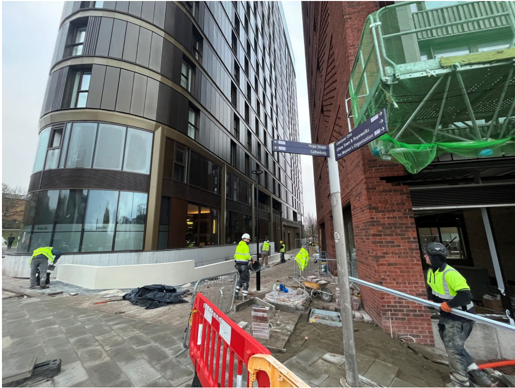
Podium paving works ongoing
