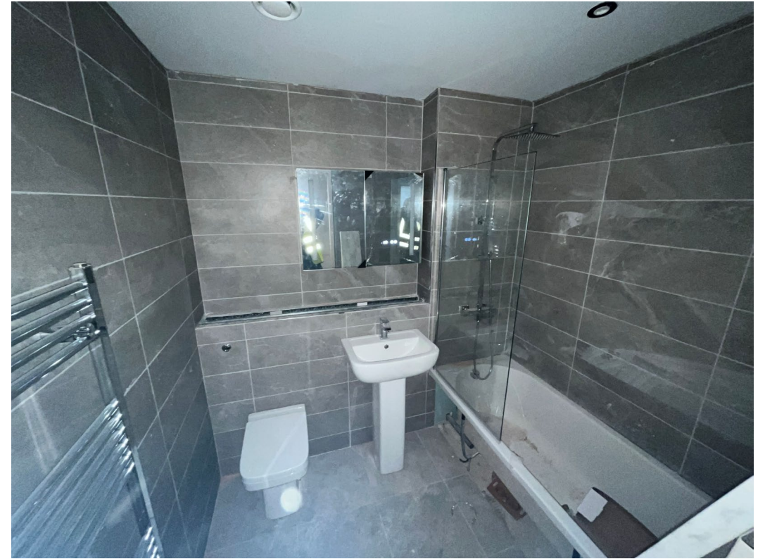
Bathroom nearing completion
