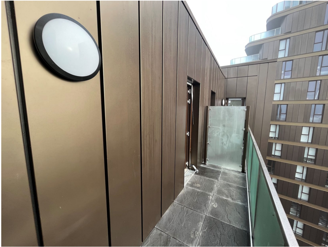
Balcony dividers installed
