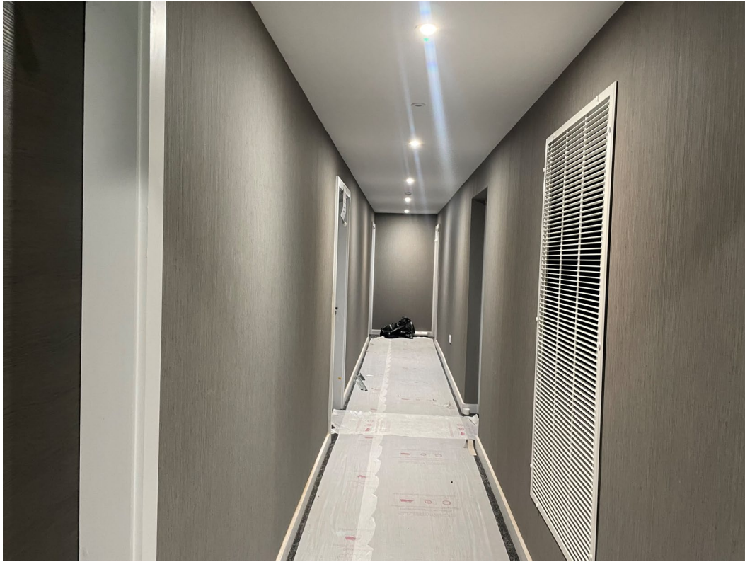
Wall coverings installed to circulation area
