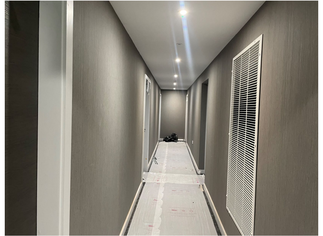
Wall coverings installed to circulation area
