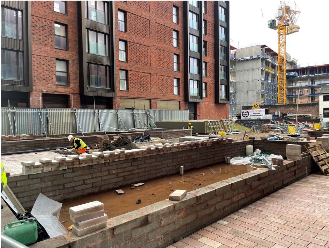
Podium works ongoing
