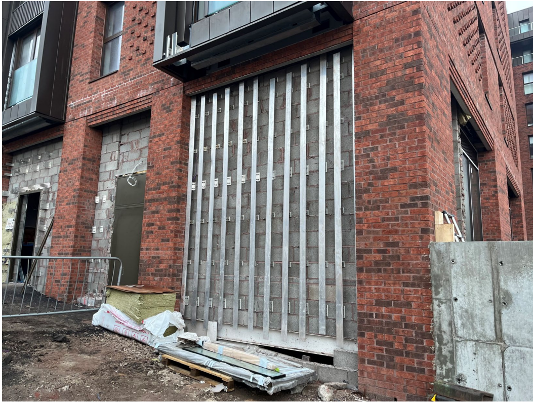
Cladding installation nearing completion
