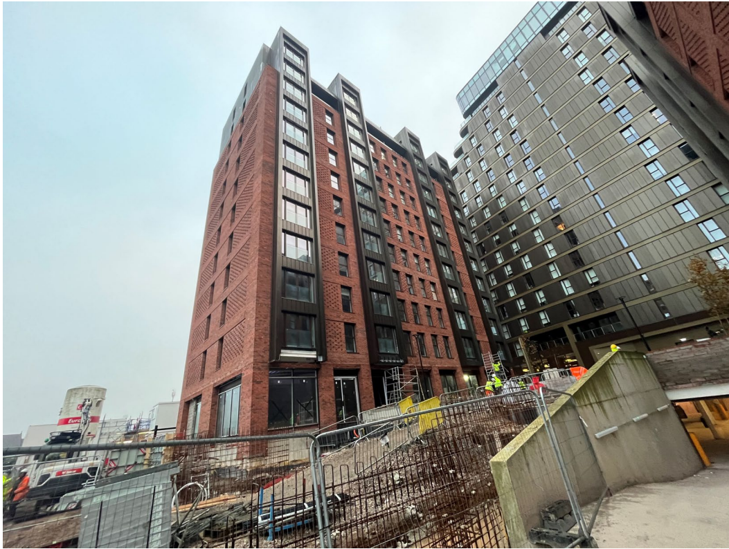
Brickwork façade nearing completion
