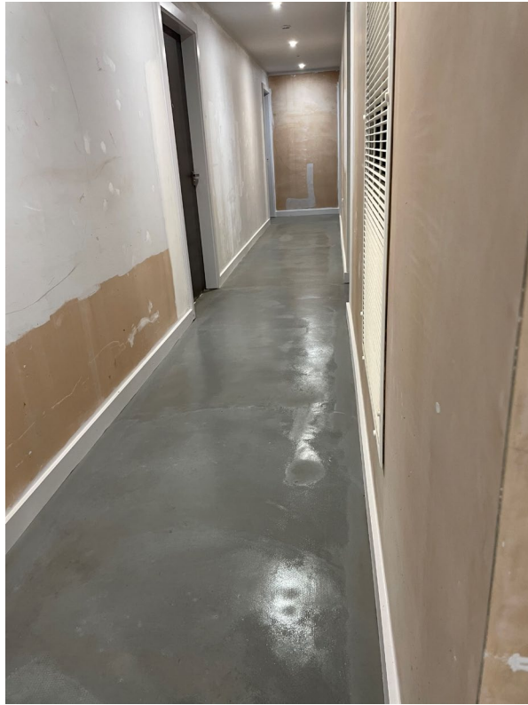
Floor screed applied to circulation areas
