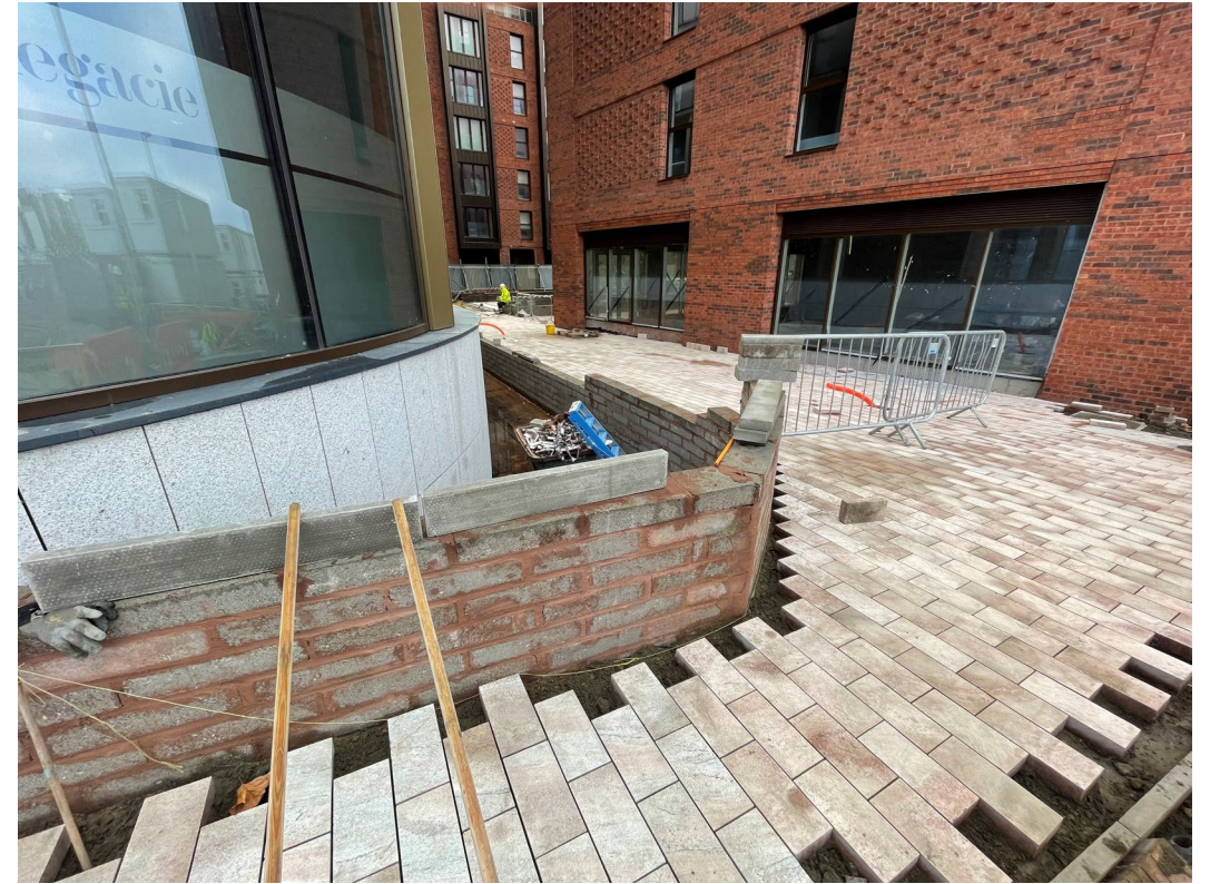
Paving works ongoing
