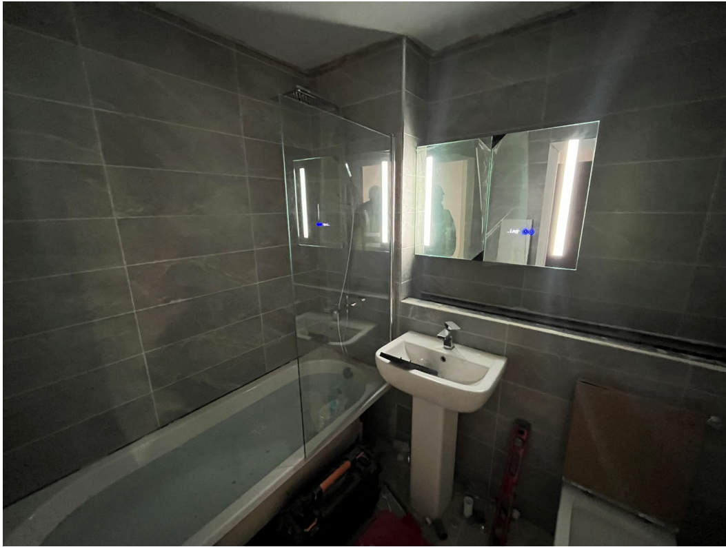
Bathroom nearing completion
