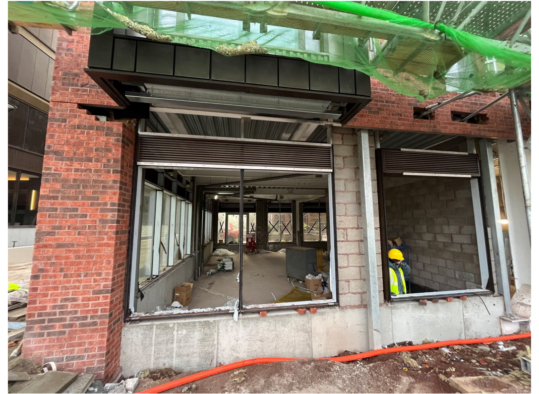
Curtain wall installation nearing completion
