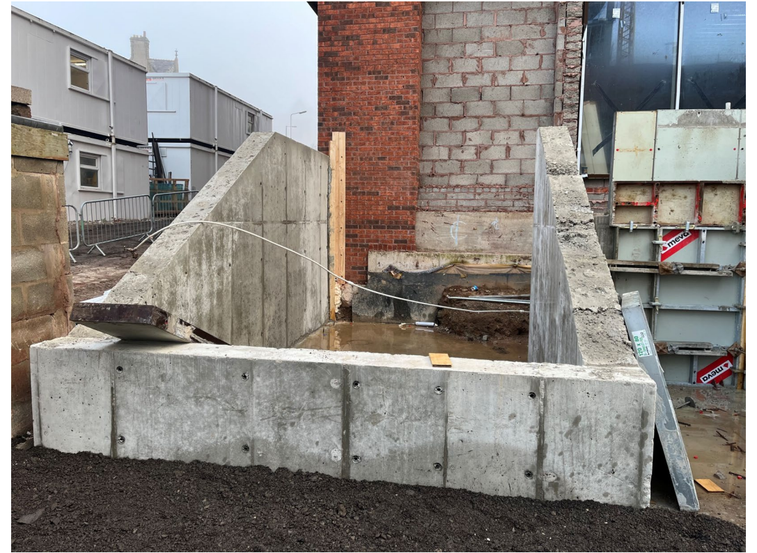
Retaining wall formed
