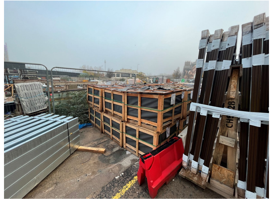
Steps on site for installation
