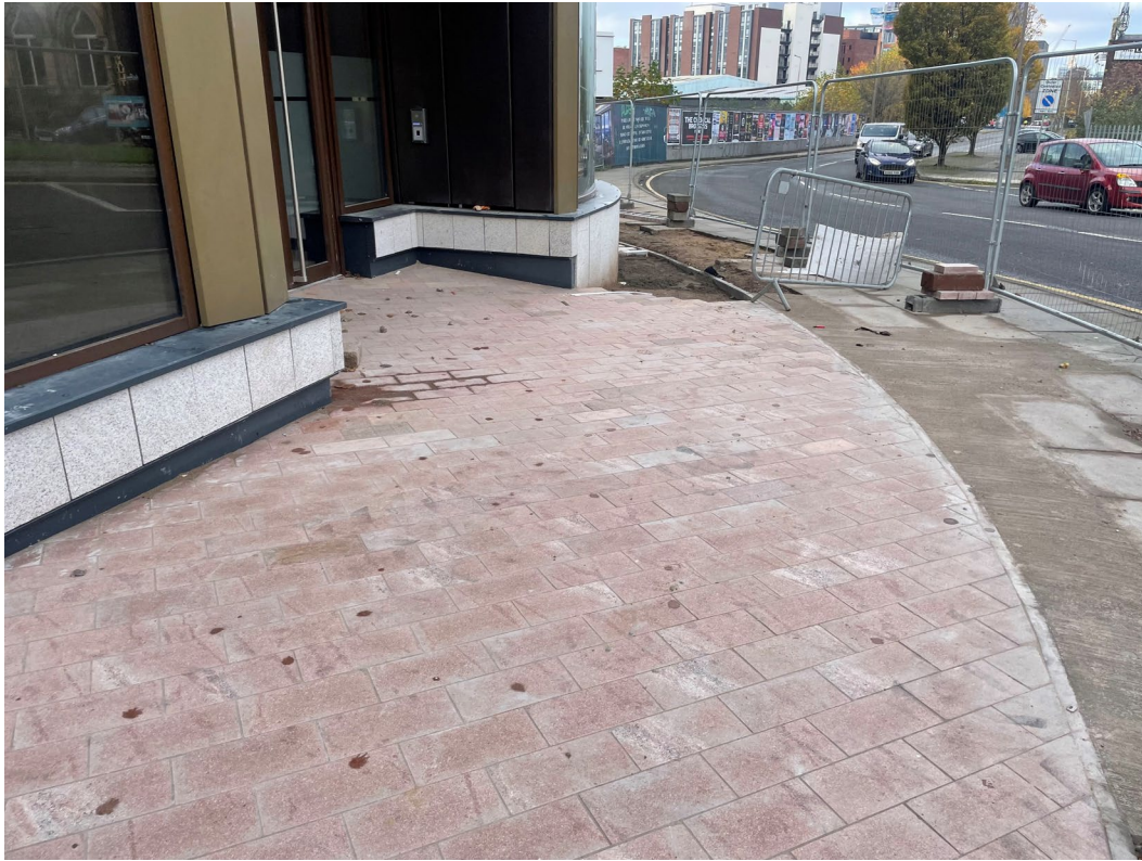
Paving works ongoing
