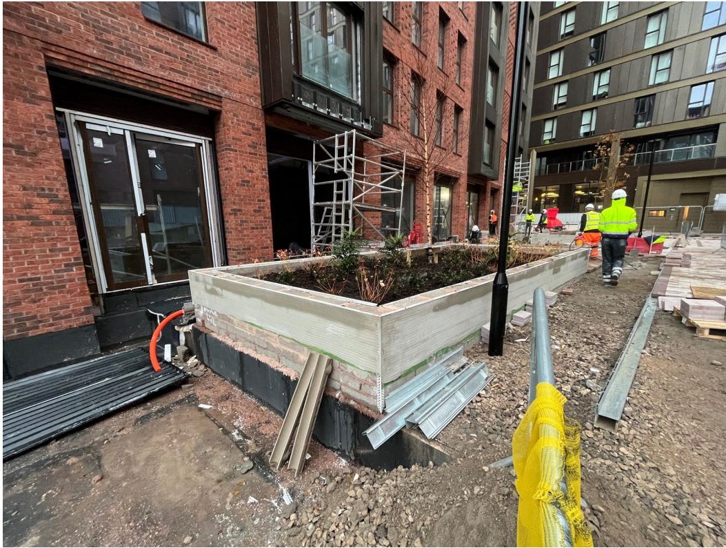
Raised planted ready for render application
