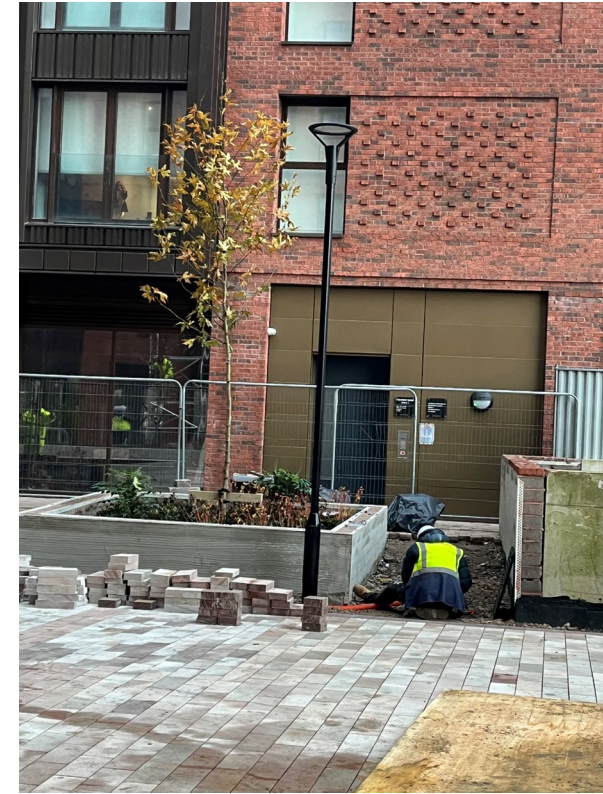
Street light installed
