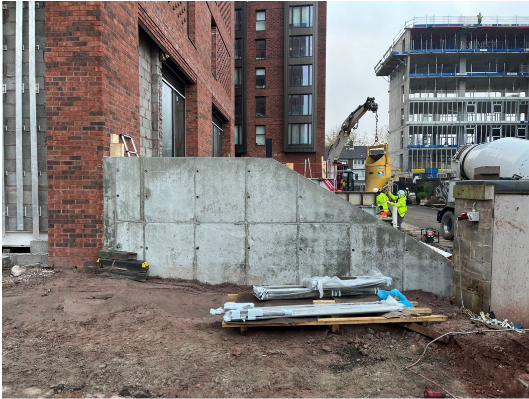
Retaining wall formed
