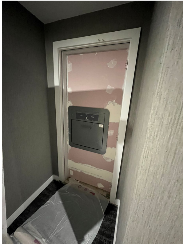
Bin chute installed
