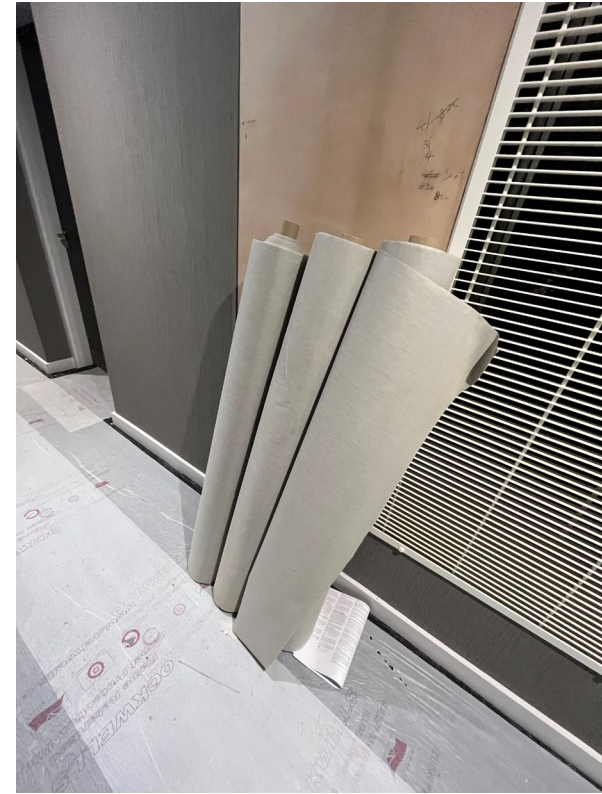
Wall coverings ready for installation
