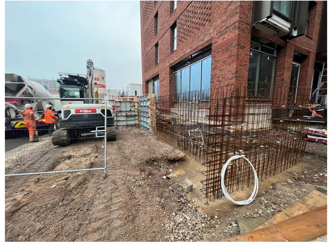
Formwork and reinforcement for retaining walls
