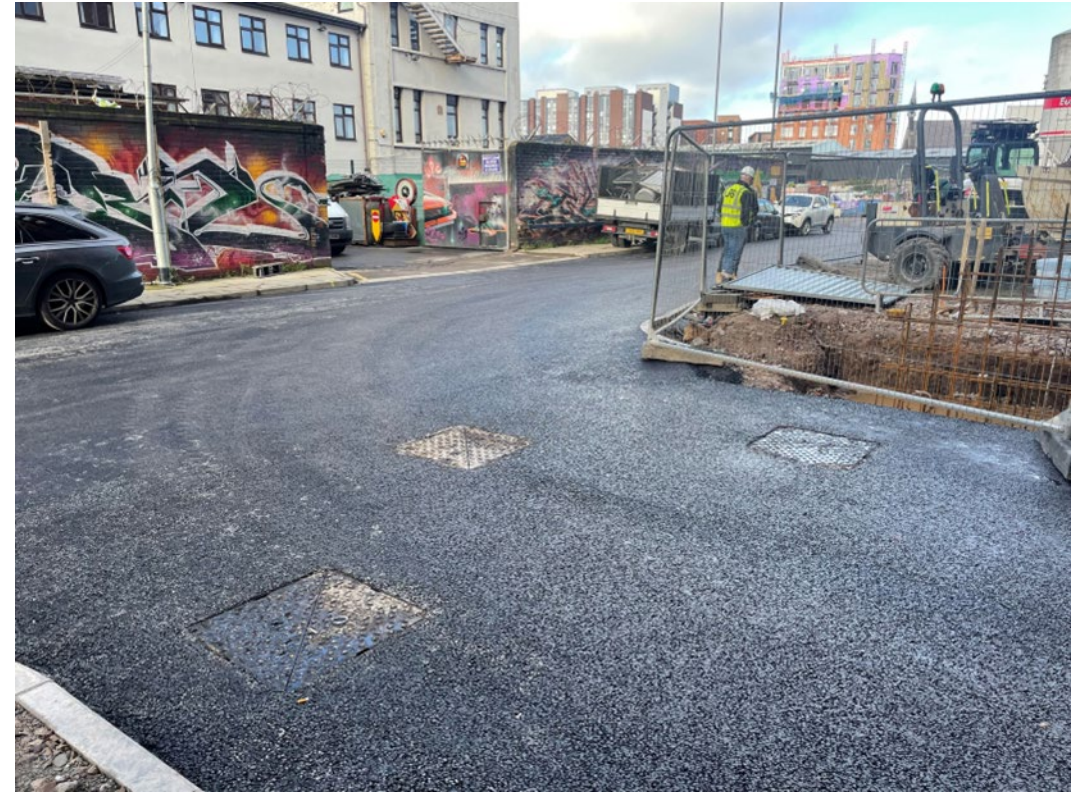
Temporary tarmac topcoat installed for basement access
