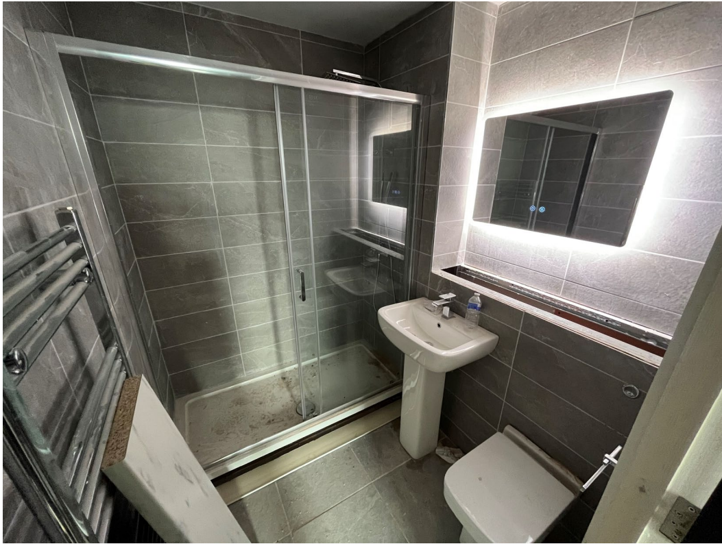
En-suite installation nearing completion
