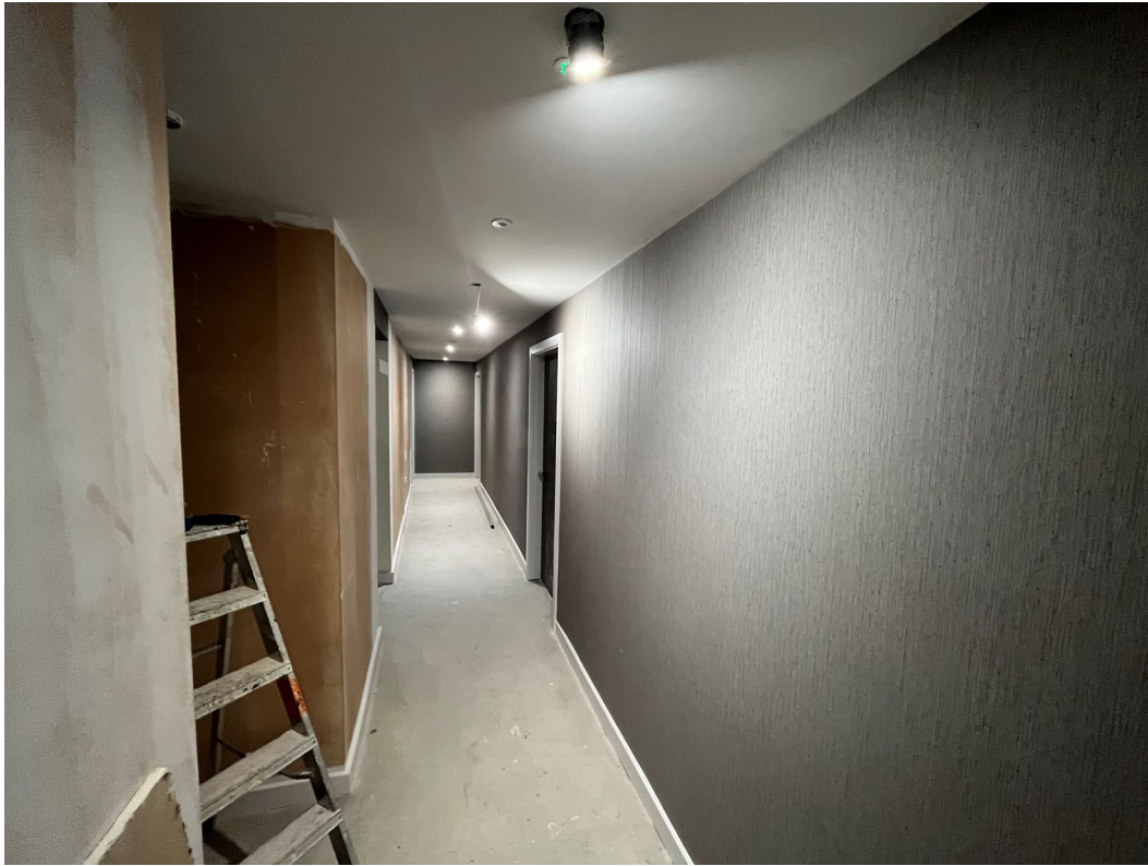
Wall coverings installed to circulation area
