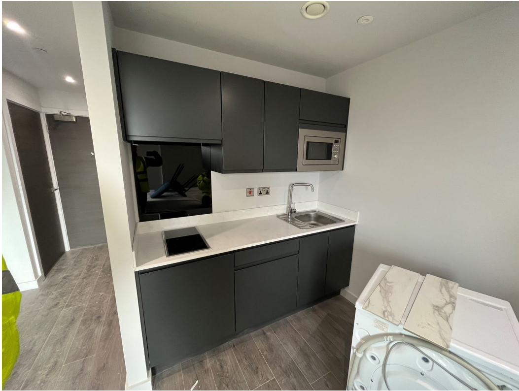
Kitchen installation complete
