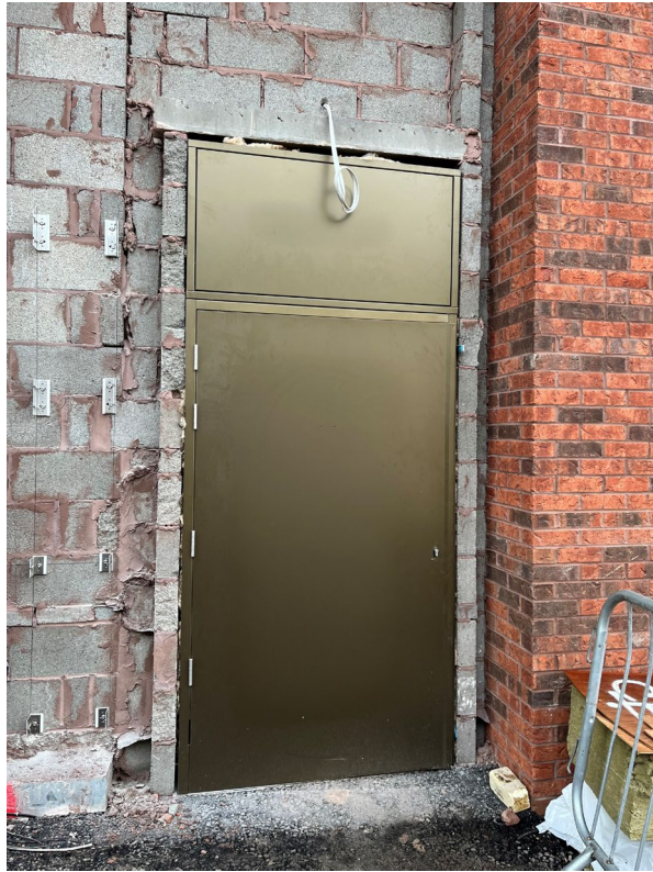
External door installed
