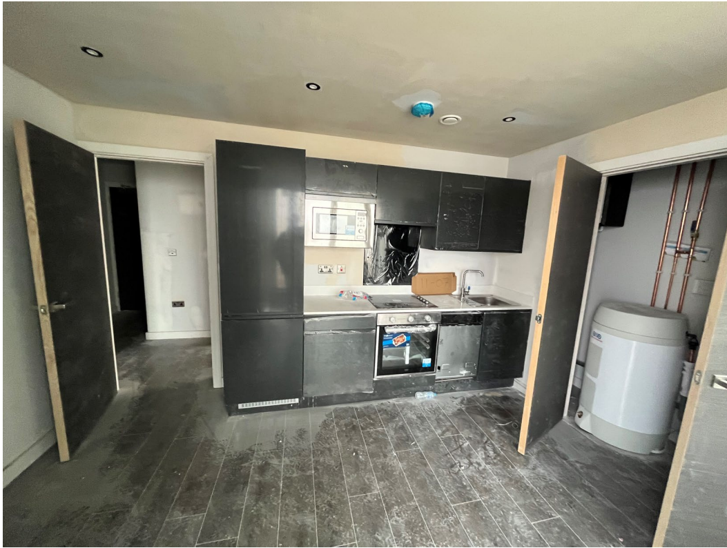
Kitchen installation nearing completion
