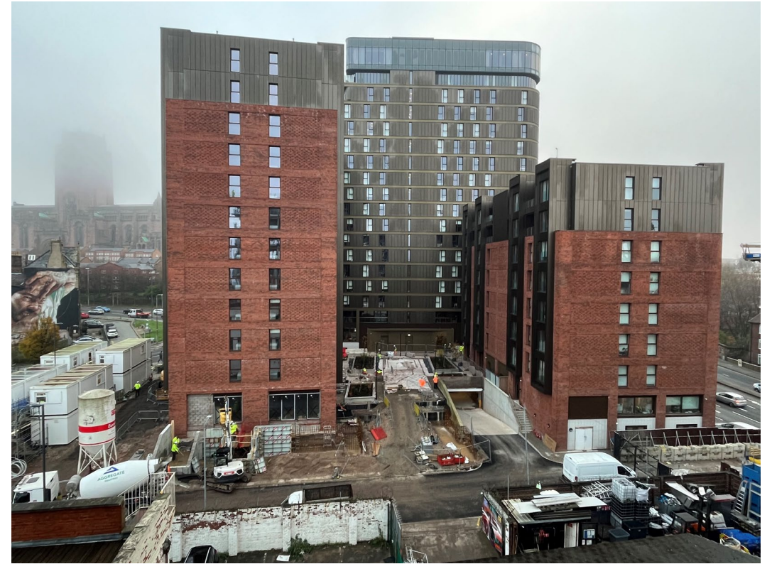
Block B – Viewed from Block D
