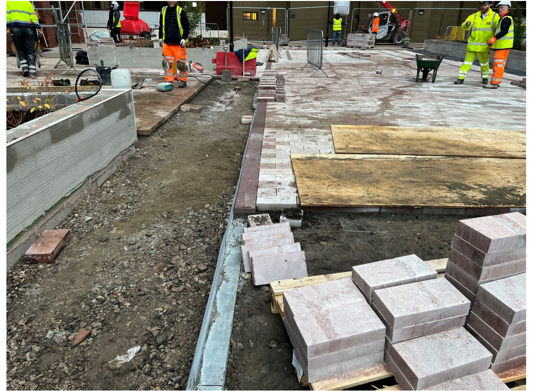
ACO Slimline Drains installed
