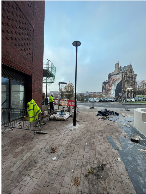
Street light installed
