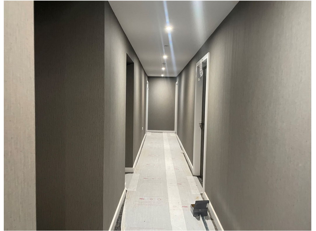
Wall coverings installed to circulation area
