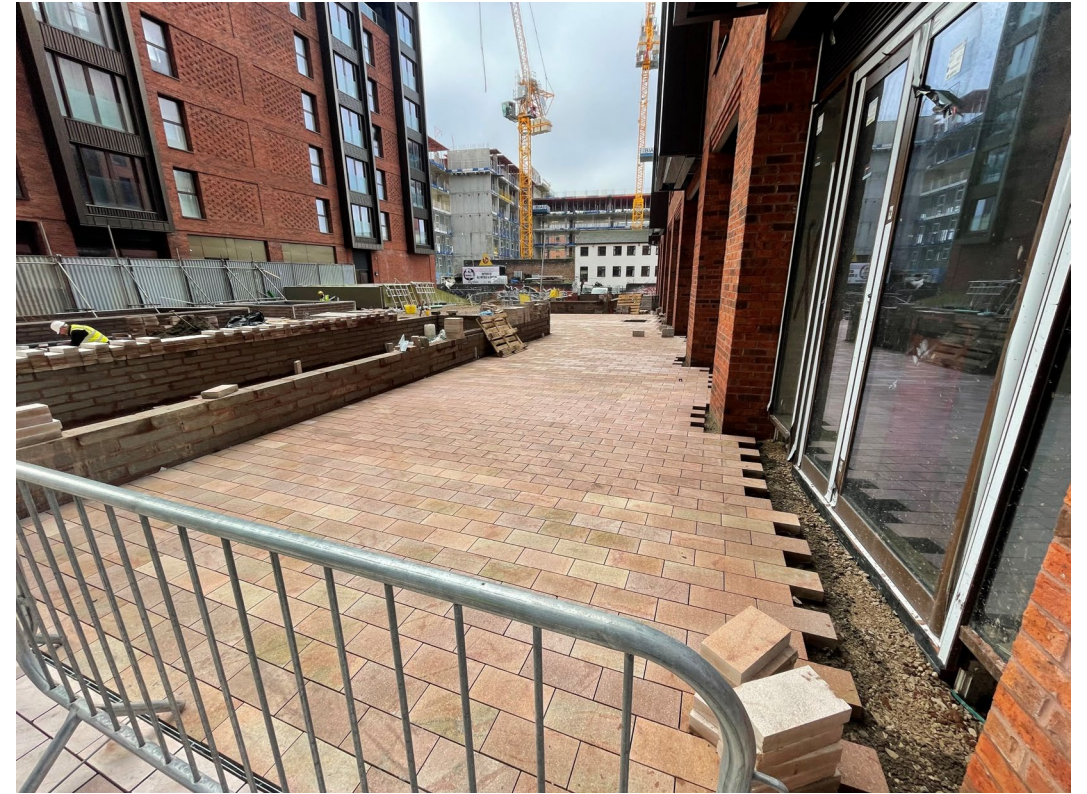
Paving works ongoing
