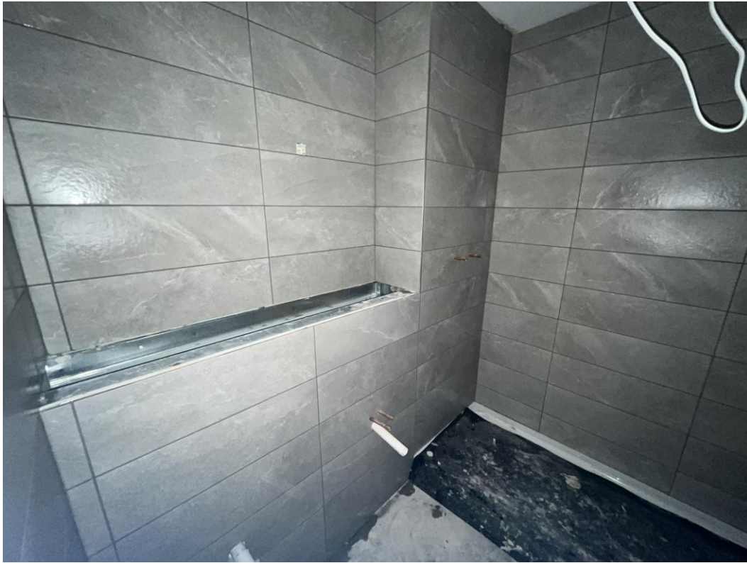
Pattress installation and IPS ongoing
