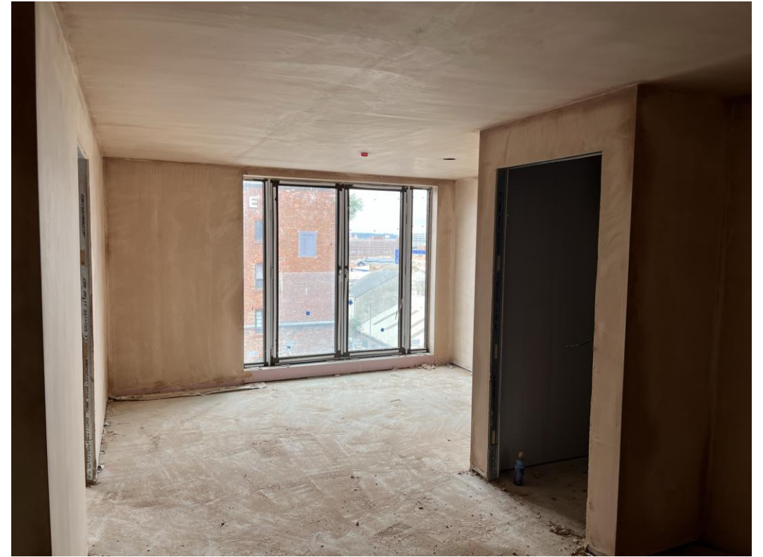
Plaster skim walls and ceiling application ongoing
