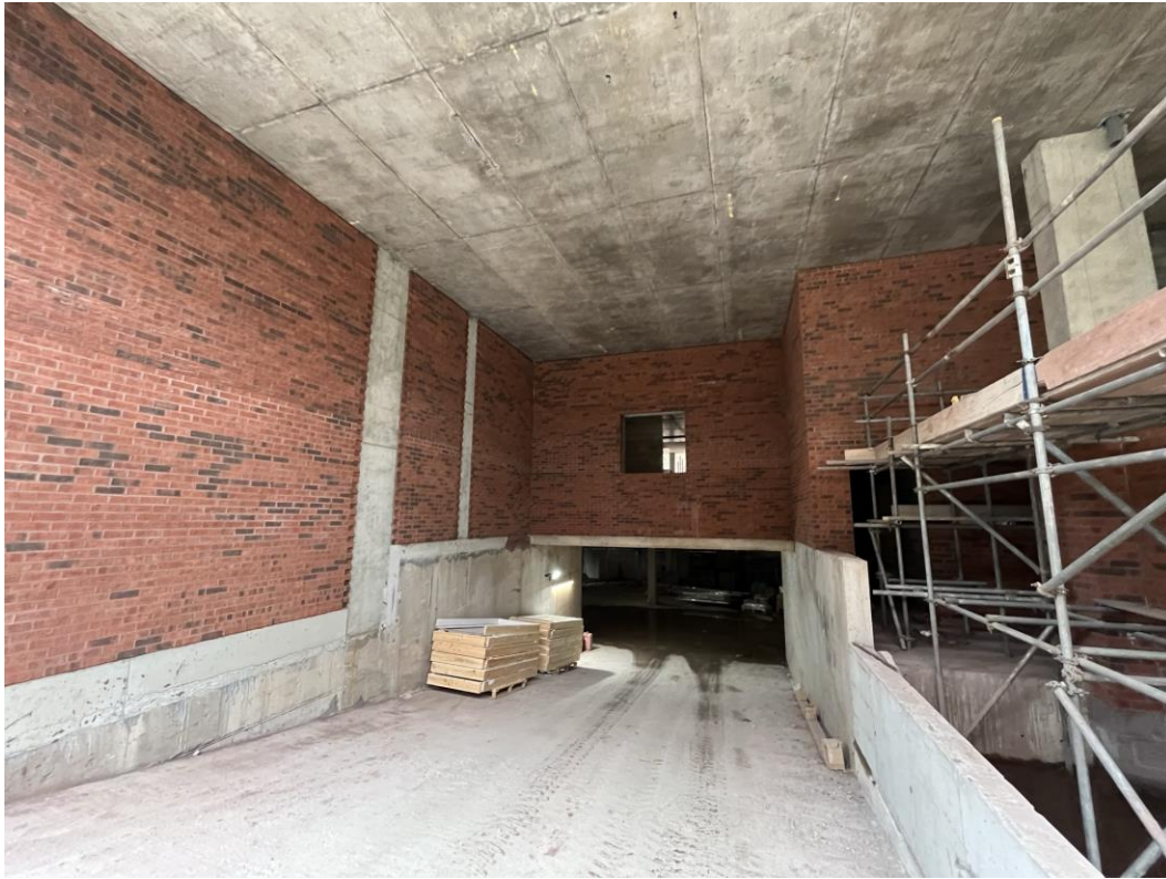
Ground floor brickwork ongoing
