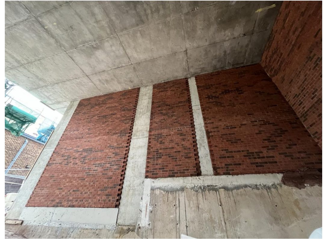
Ground floor brickwork ongoing
