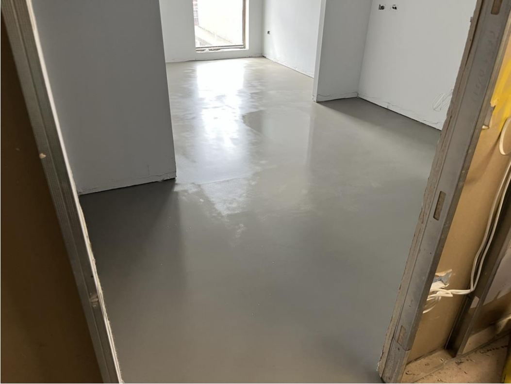
Self-levelling screed application ongoing
