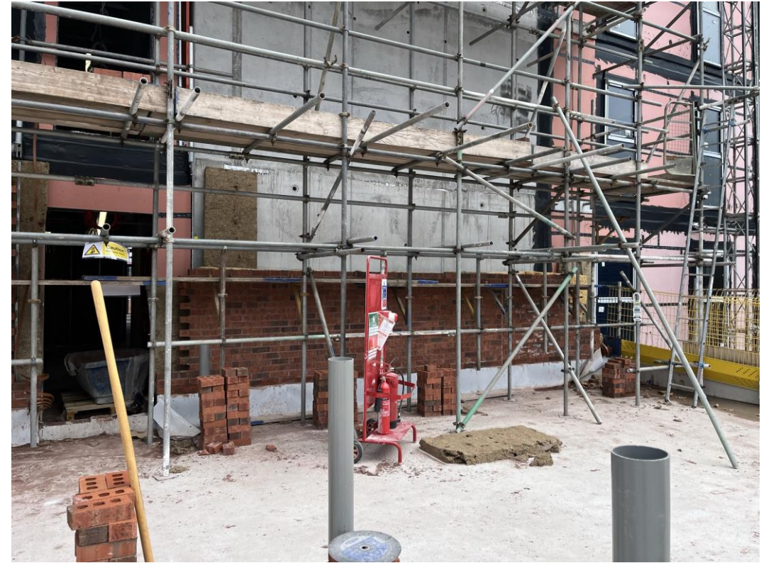
External brickwork ongoing
