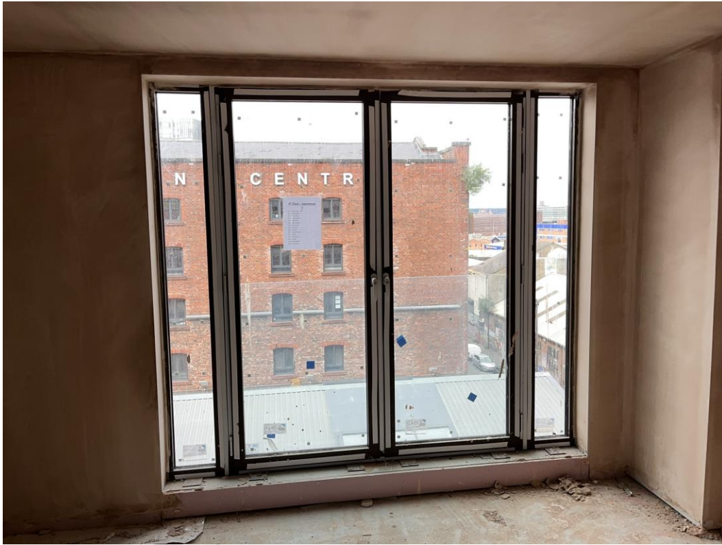
Plaster skim walls and ceiling application ongoing
