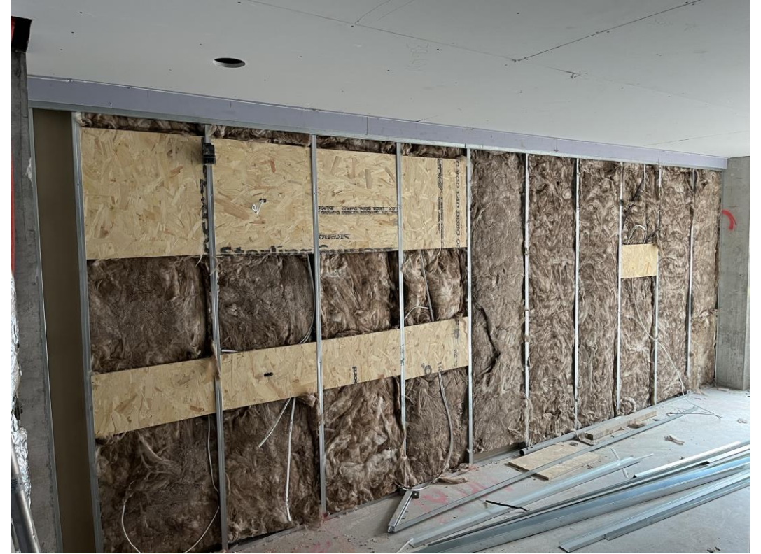
Insulation and pattress installation ongoing
