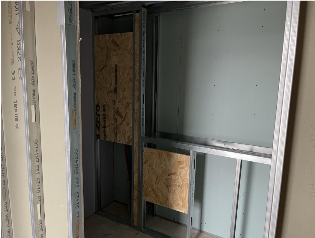
Pattress installation and IPS ongoing
