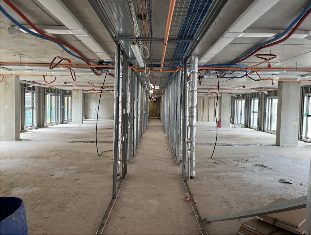
Erection of metal partition walls ongoing
