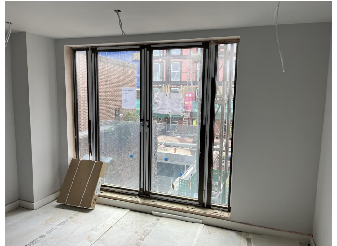
Mistcoat application ongoing
