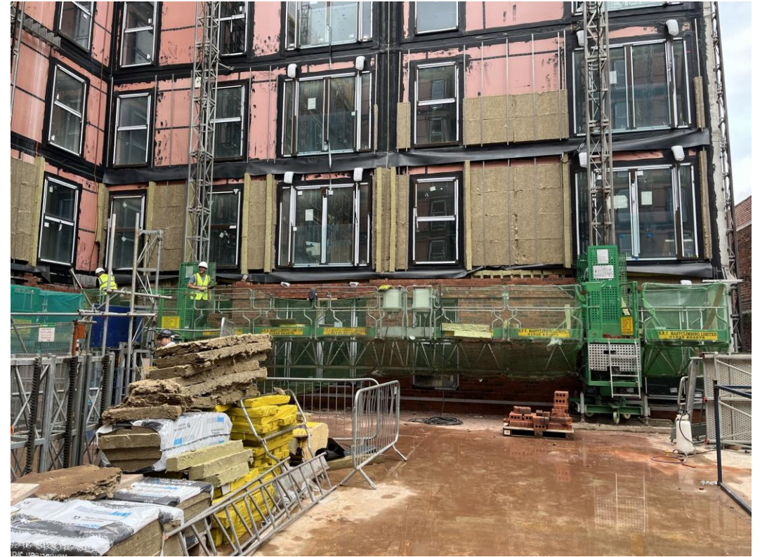
Block D Section A – Mast climbers
