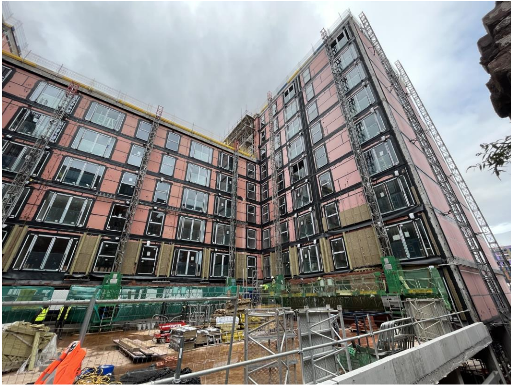
Block D Section A – Mast climbers
