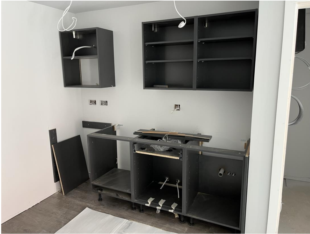
Installation of kitchen units ongoing
