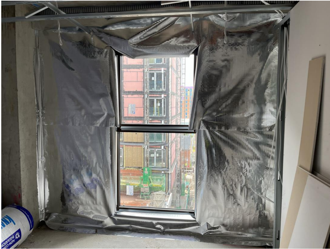
Insulating of external walls ongoing
