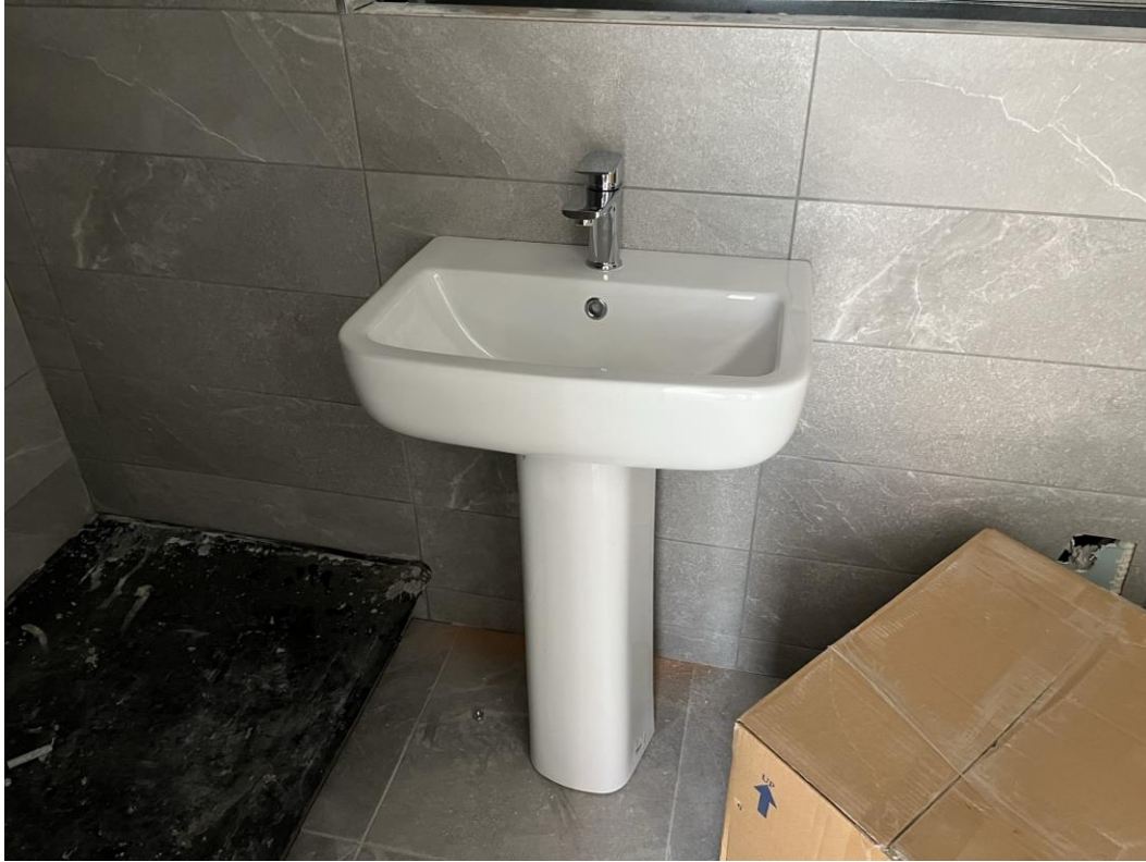
Sanitaryware installation ongoing
