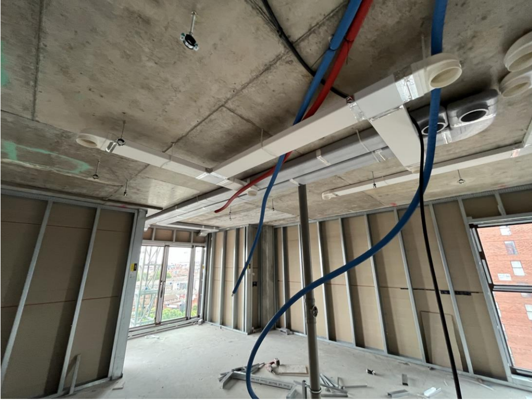
1 st fix mechanical ductwork installation ongoing
