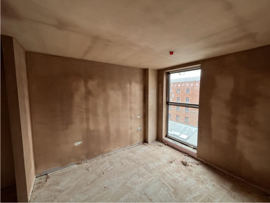
Plaster skim walls and ceiling application ongoing
