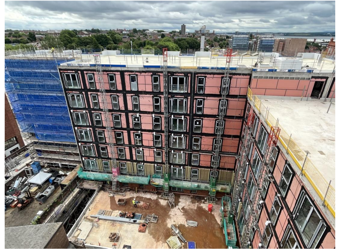
Block D Section B – SFS & Weatherboarding Installation
