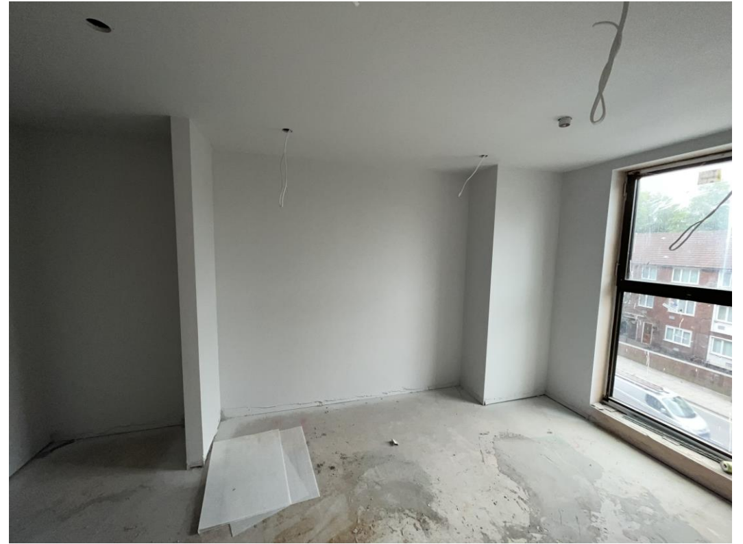
Internal finishes ongoing
