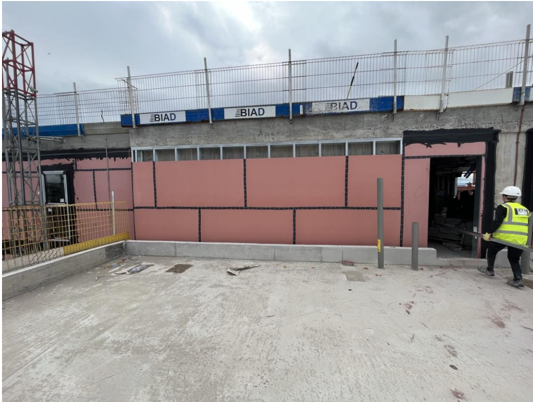
Block D – SFS & Weatherboarding installation
