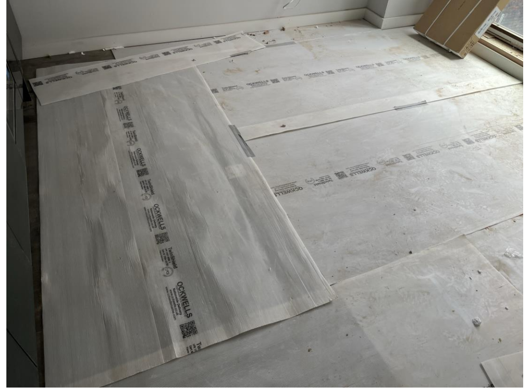
Timber flooring installation and protection ongoing
