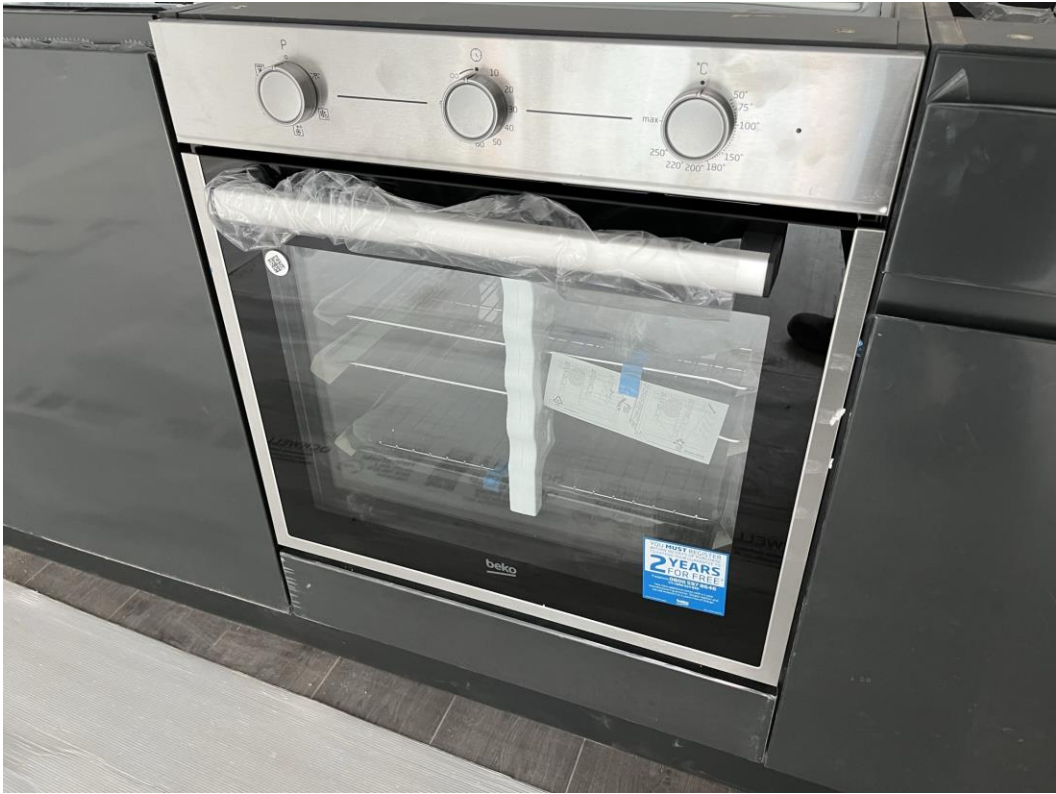
Installation of kitchen appliances ongoing
