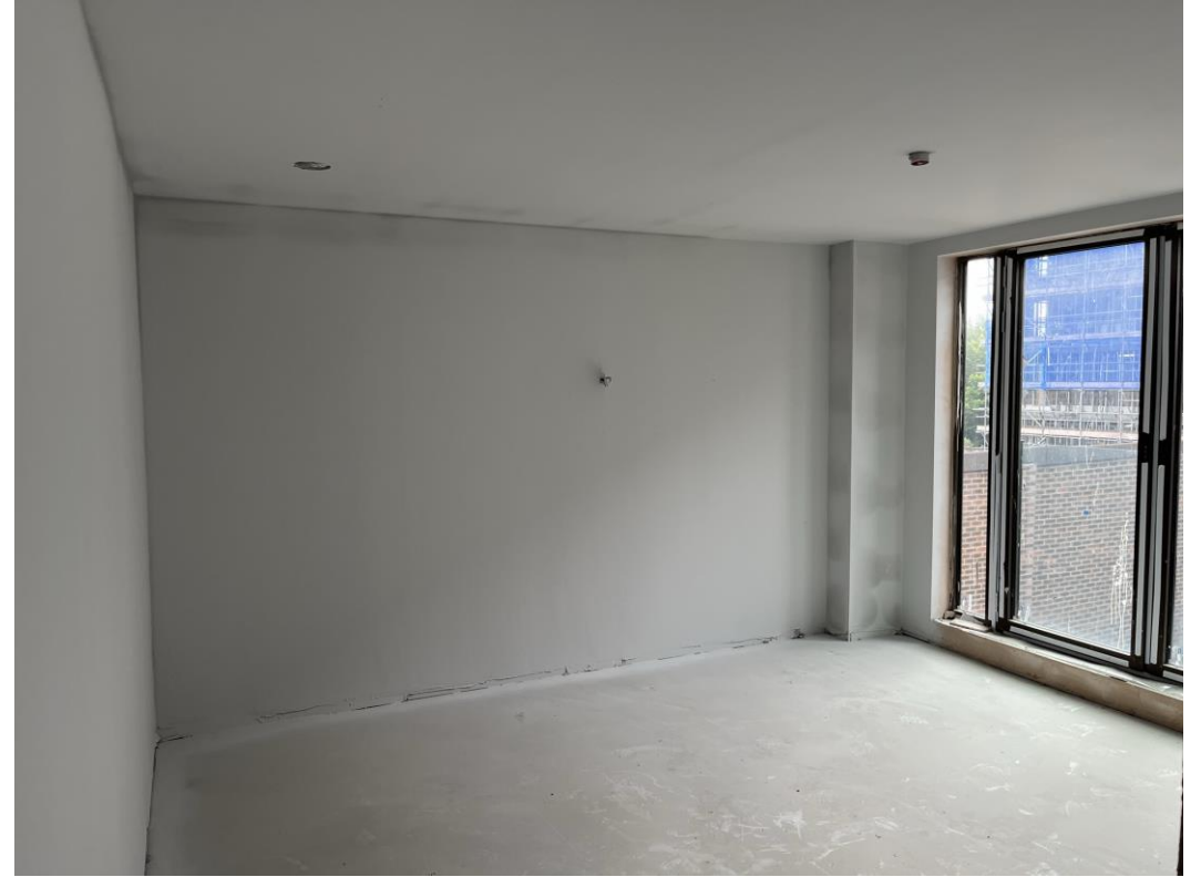
Walls and ceiling mistcoat application
