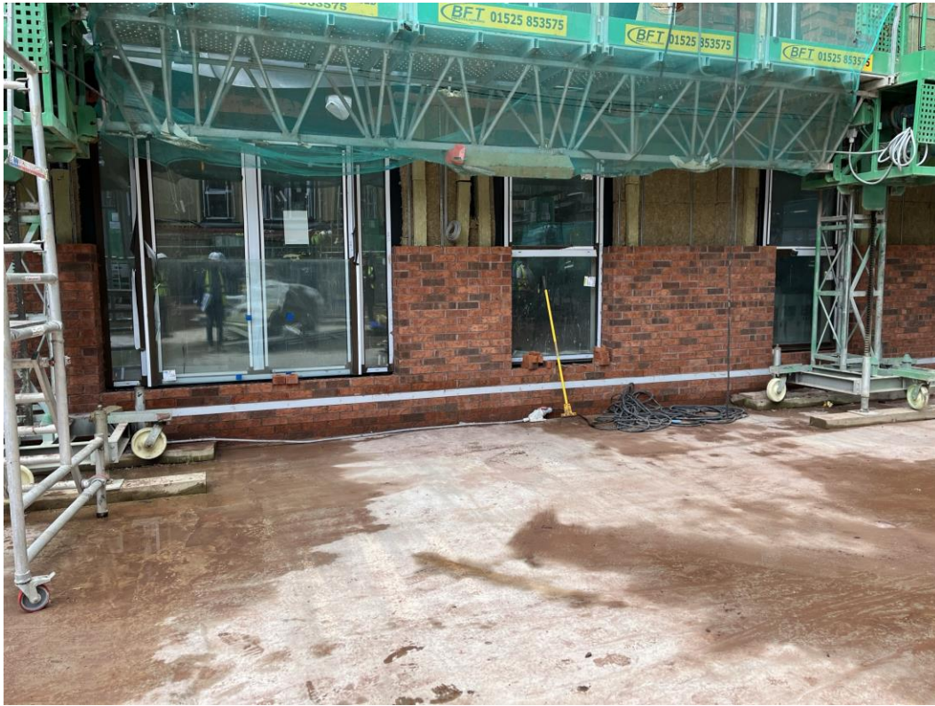
External brickwork ongoing
