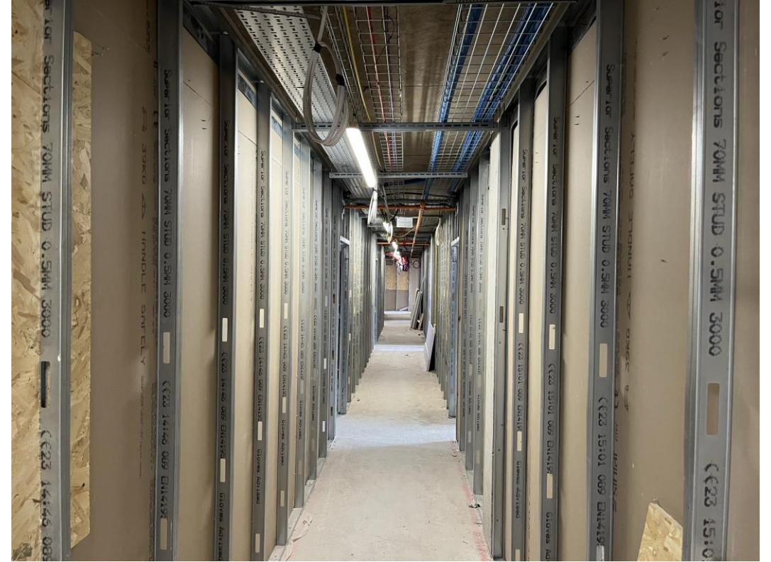
1 st side boarding of walls and pattrness installation ongoing
