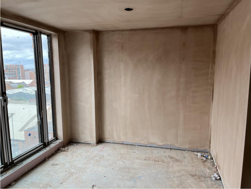
Plaster skim walls and ceiling application ongoing
