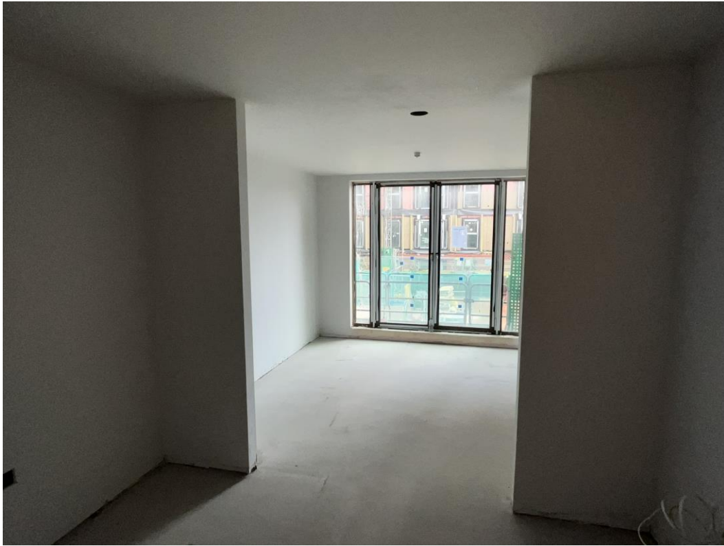
Internal finishes ongoing
