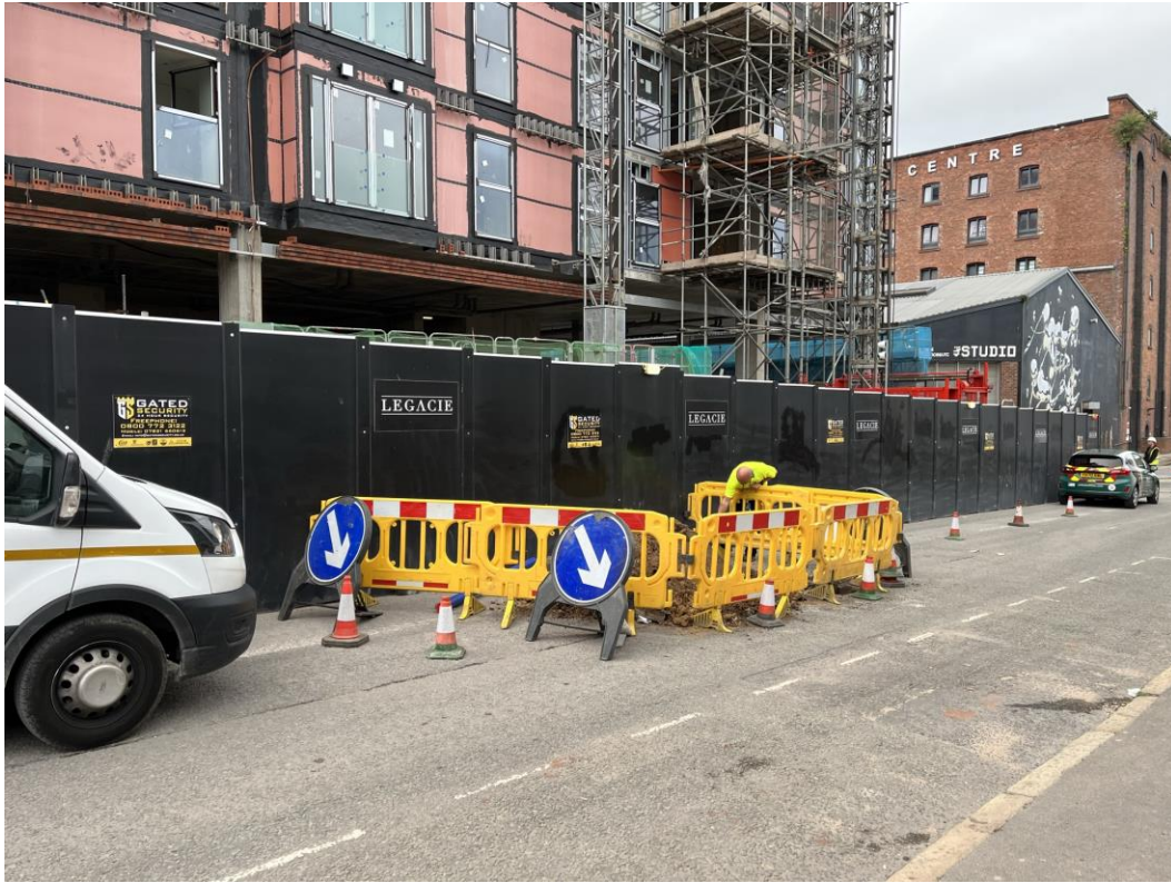
Block D Section A – Installation of underground water mains
