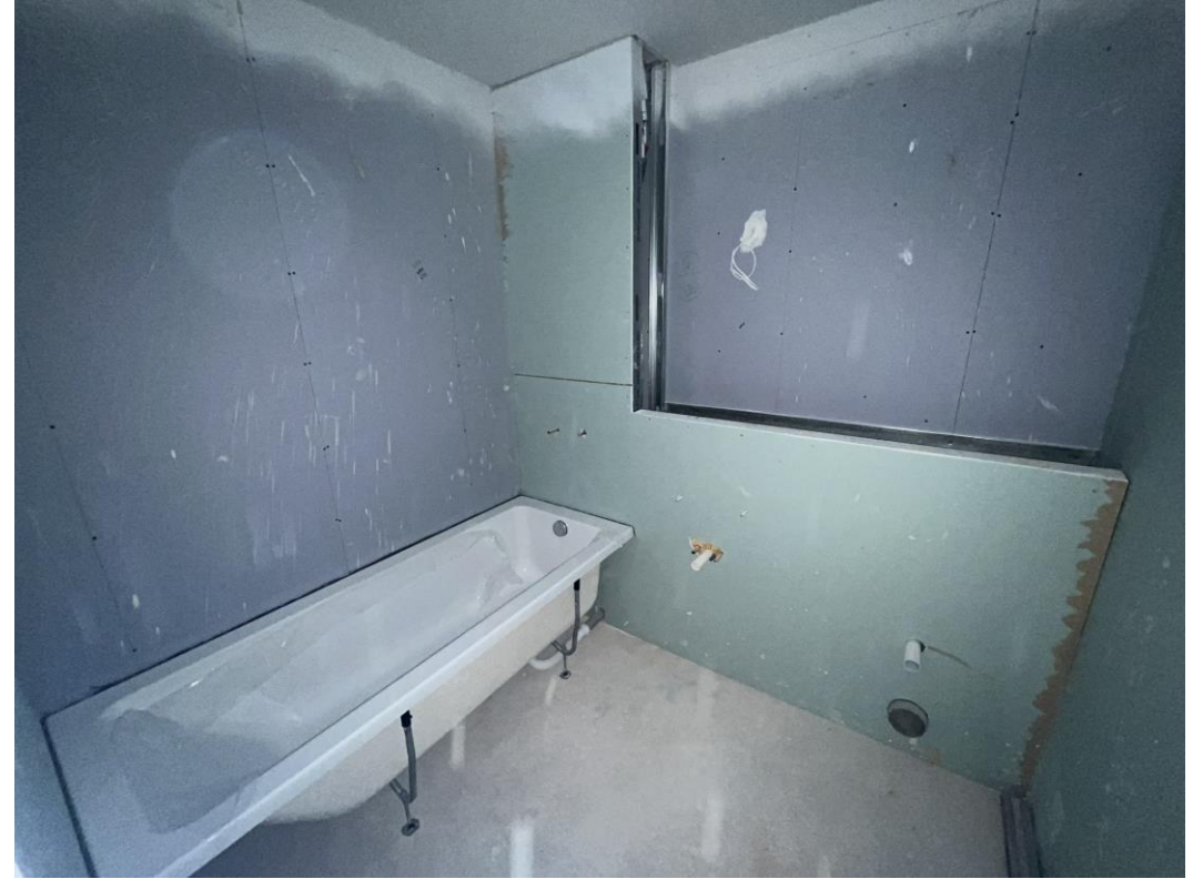
Sanitaryware installation ongoing
