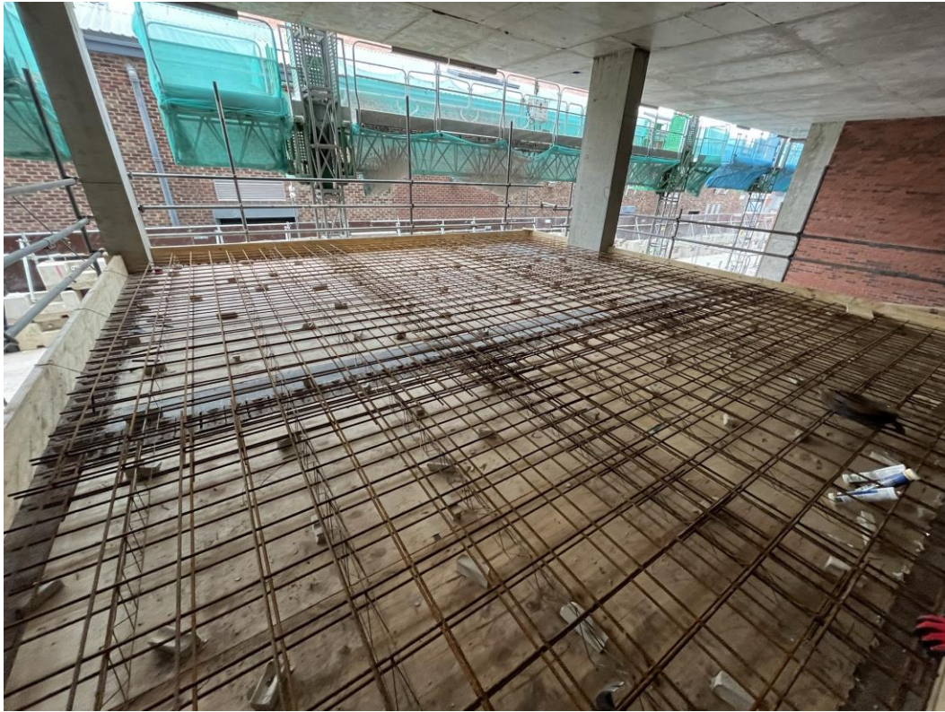
Formation of substation roof ongoing
