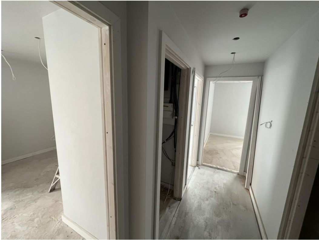
Internal joinery and internal finishes ongoing
