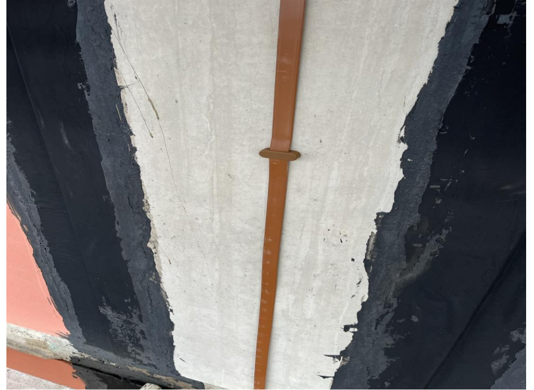
Installation of lightning protection
