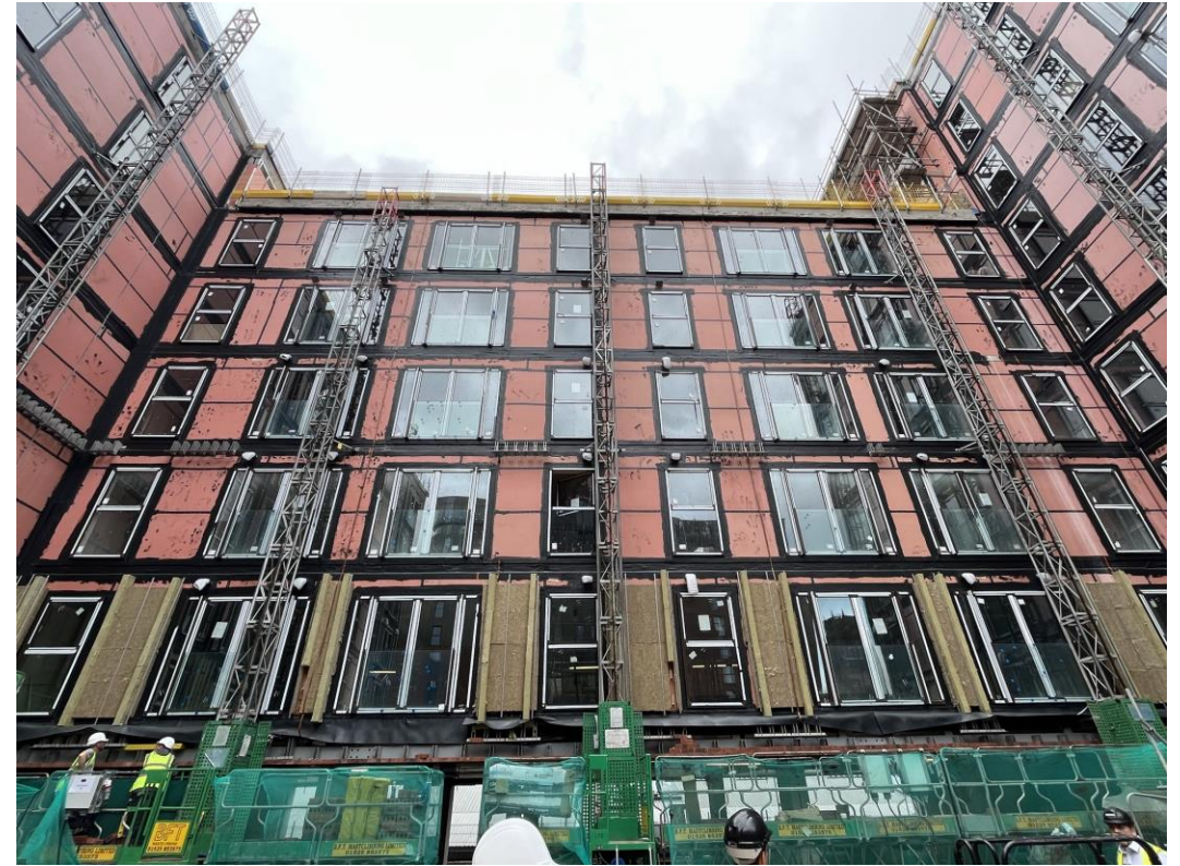
Block D Section C – Mast climbers
