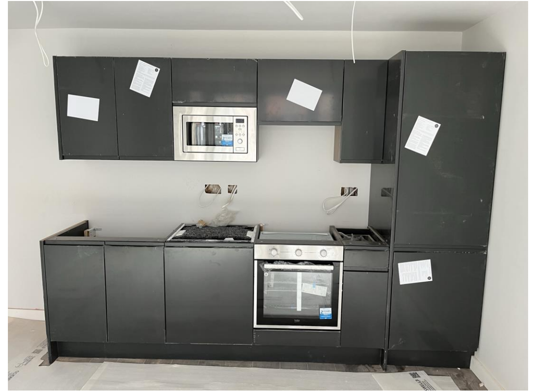
Installation of kitchen units and appliances ongoing
