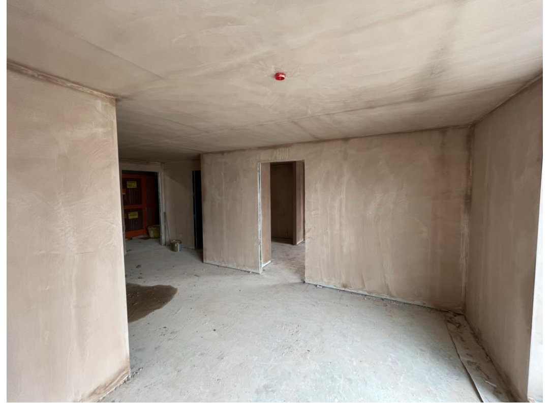
Plaster skim walls and ceiling application ongoing
