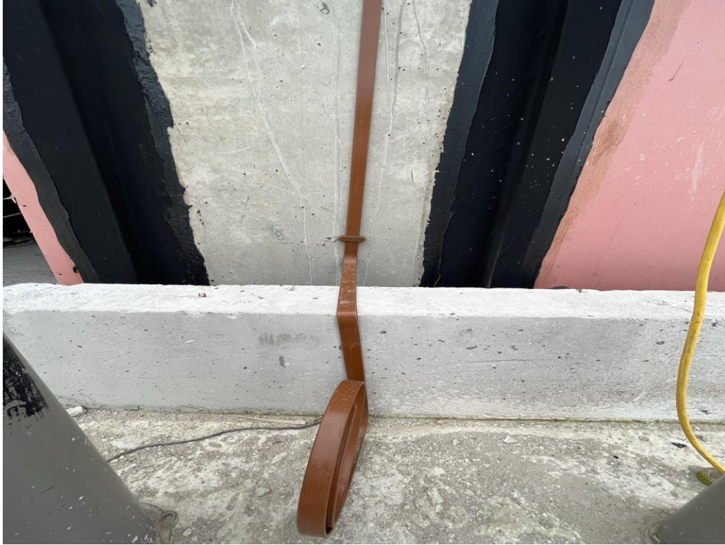
Installation of lightning protection
