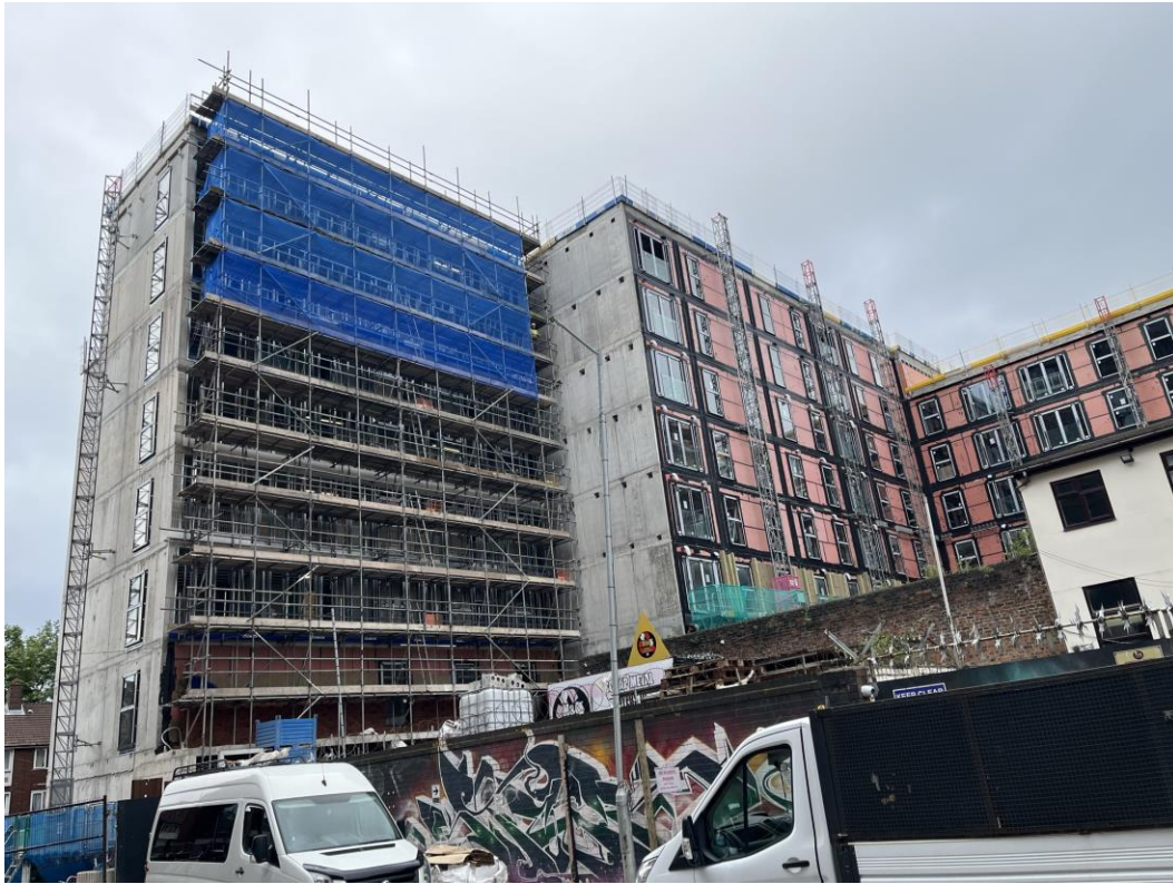
Block D Section B – Viewed from Crump Street
