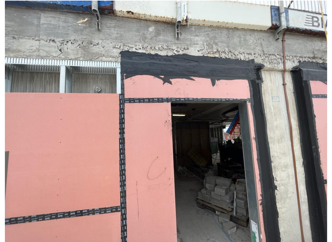
Block D – Weatherboarding and waterproofing installation
