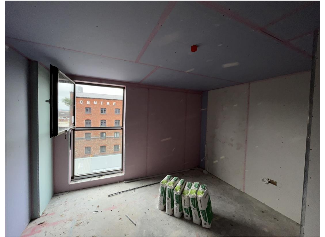
Insulating of external walls and 2 nd side boarding ongoing
