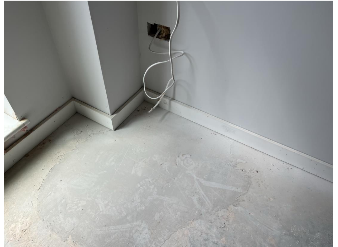
Timber skirting board installation ongoing
