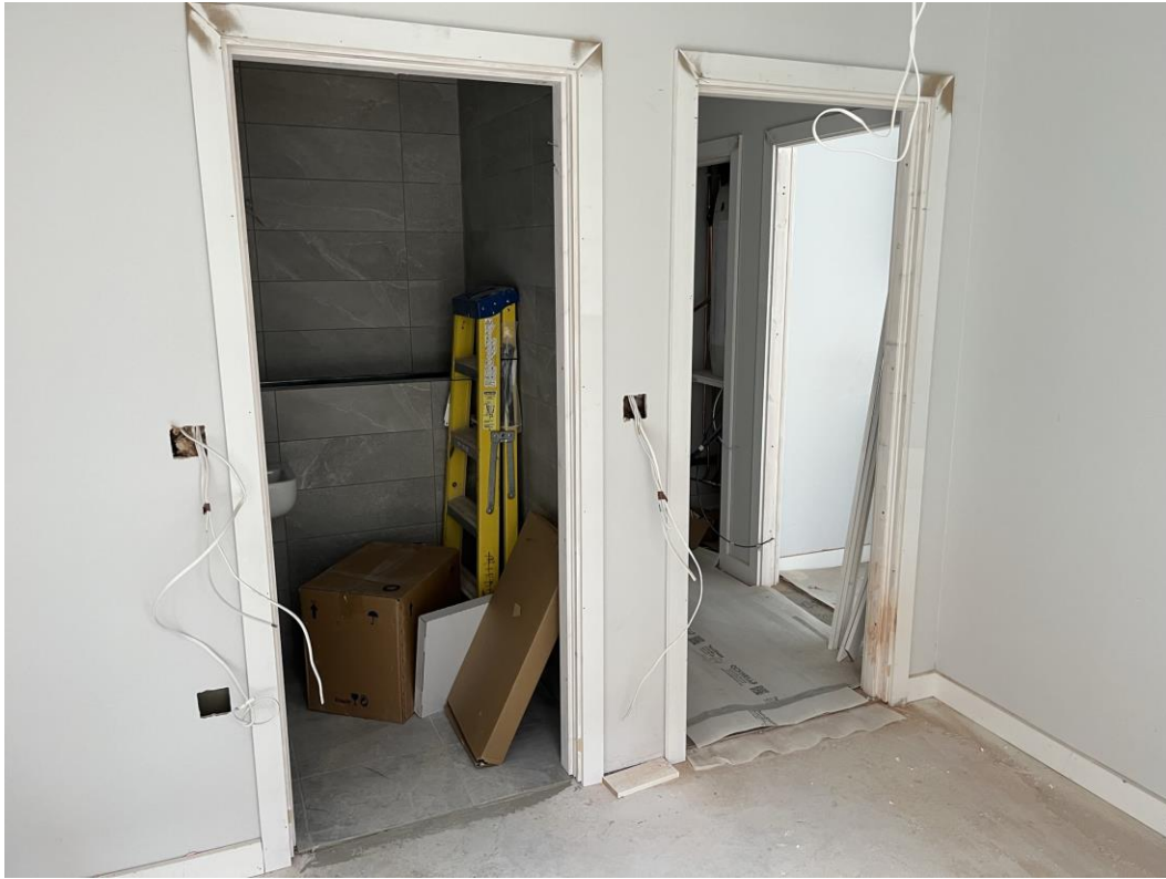
Internal joinery installation ongoing
