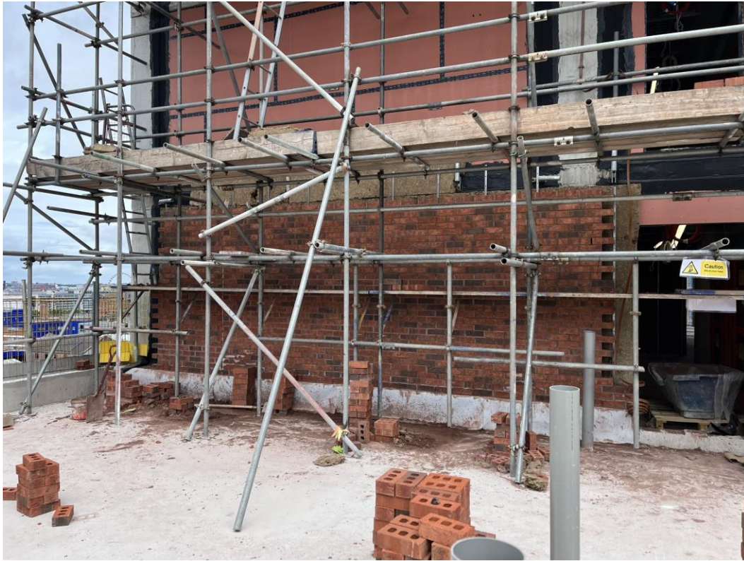
External brickwork ongoing
