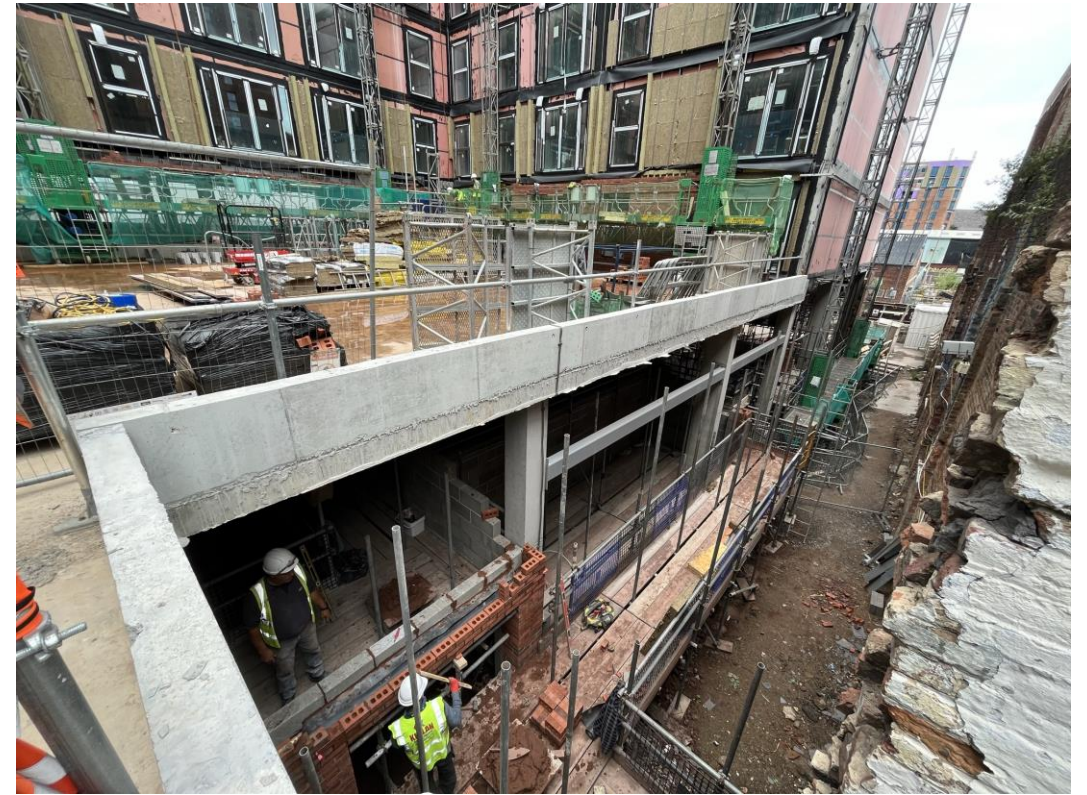
External brickwork ongoing
