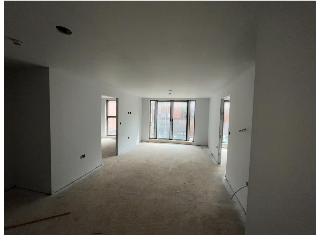
Internal finishes ongoing
