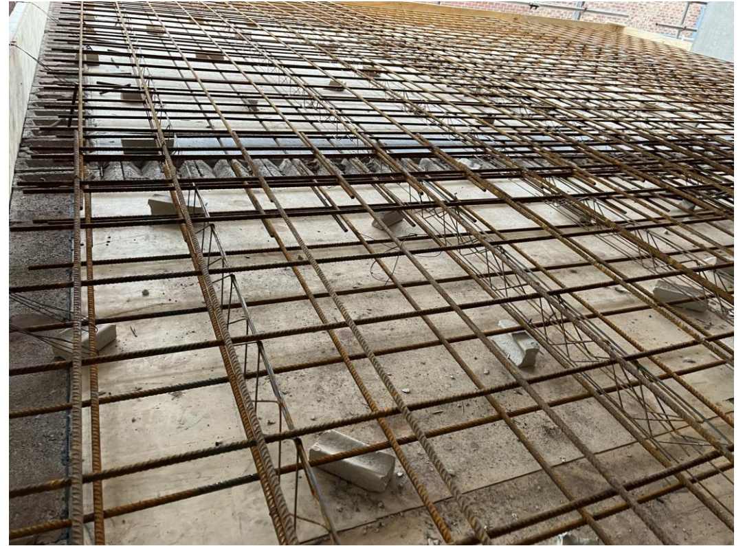
Formation of substation roof ongoing
