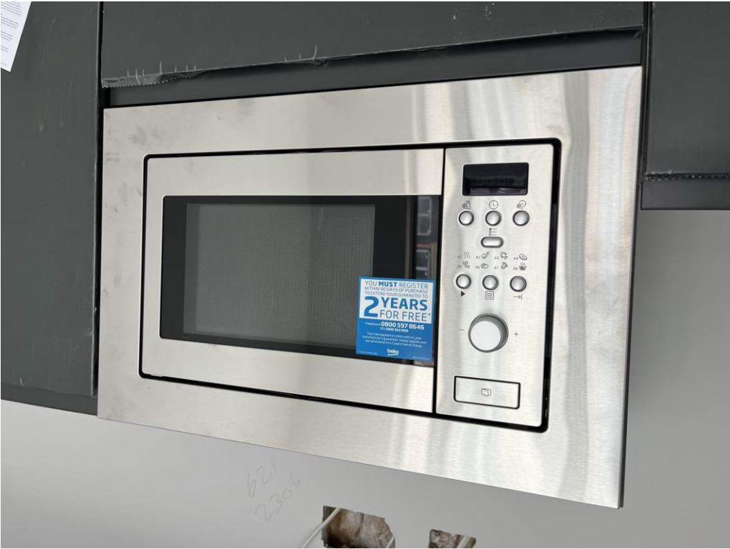
Installation of kitchen appliances ongoing
