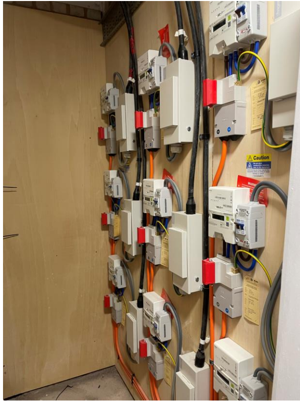
Electric meters installed
