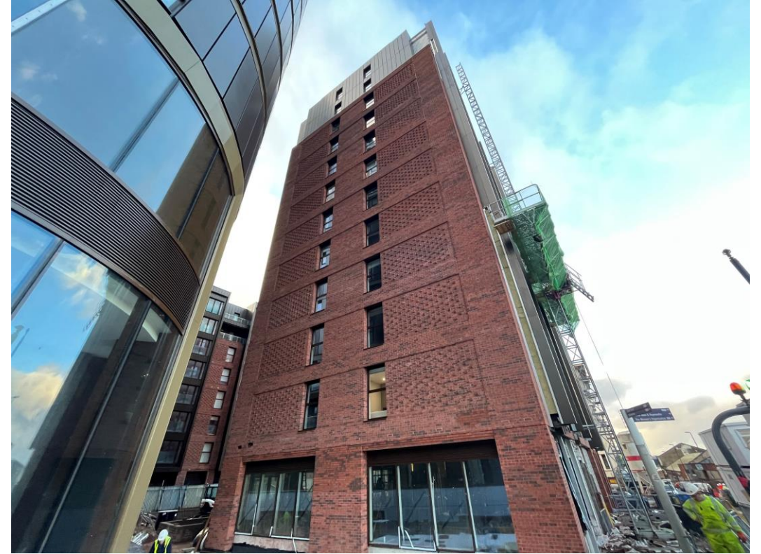
Brickwork façade nearing completion
