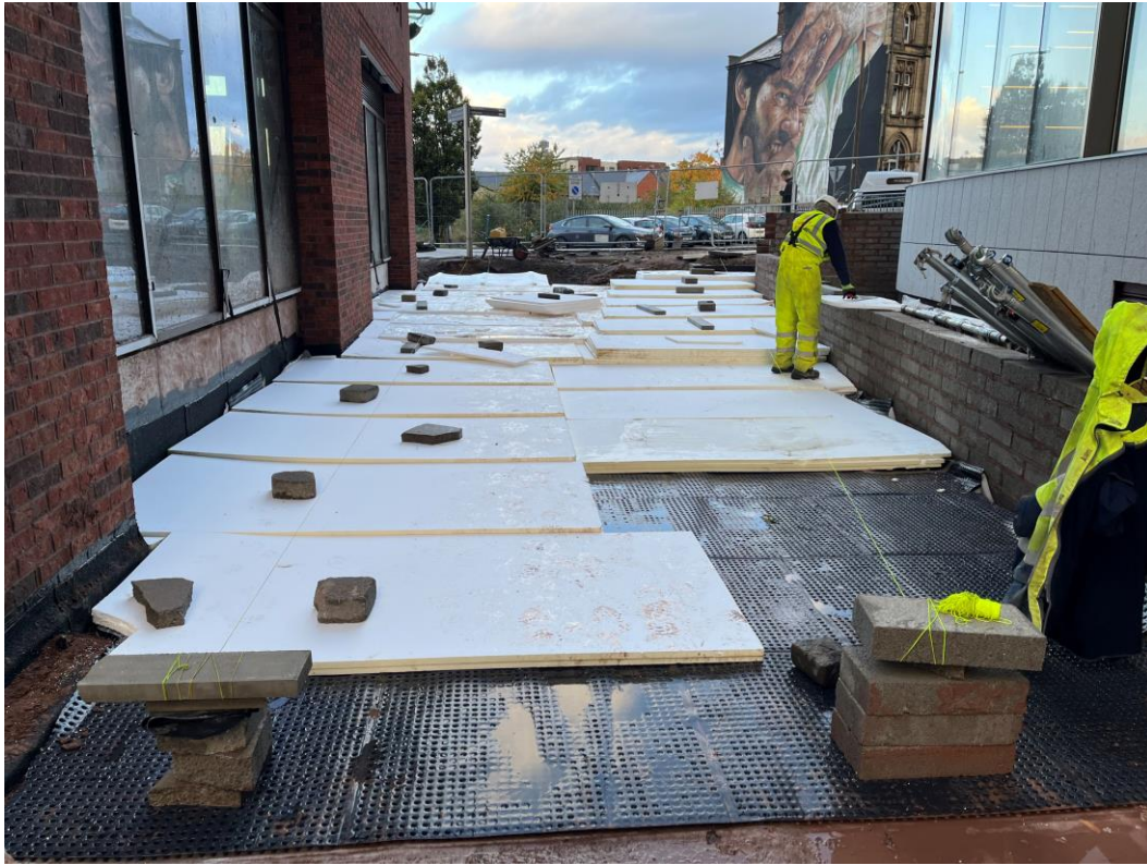
Insulation installed for podium build up
