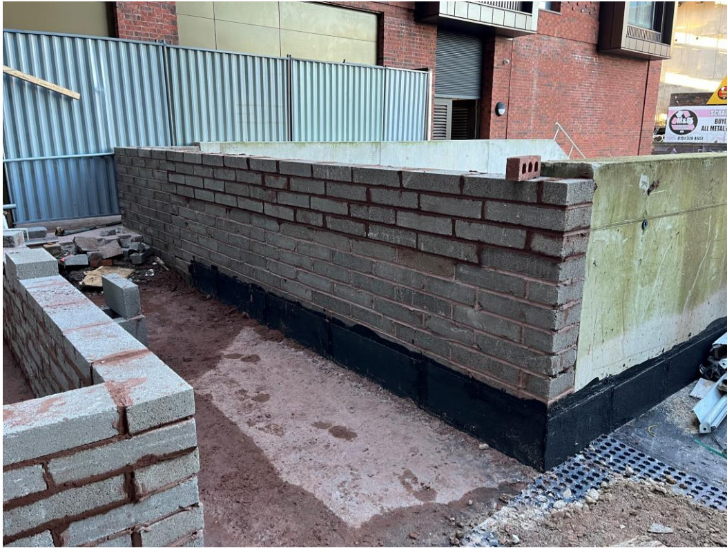
Basement access wall construction complete
