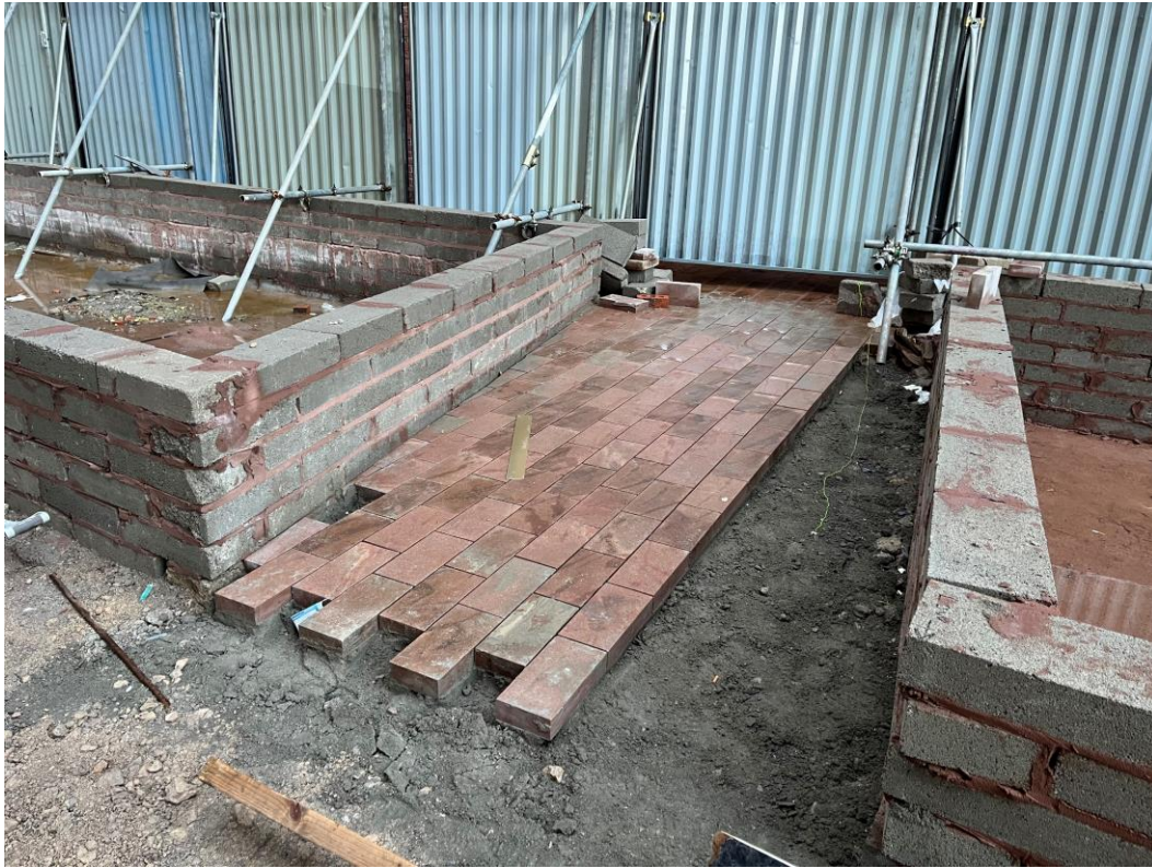
Paving flag installation ongoing
