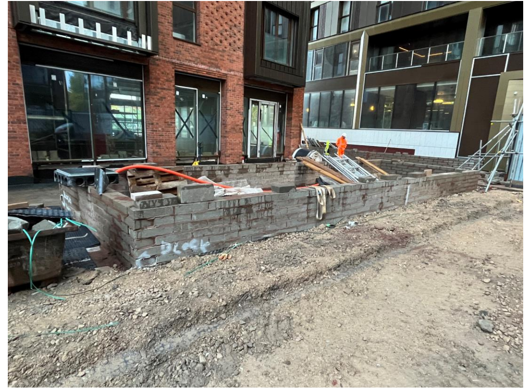
Raised planter construction ongoing
