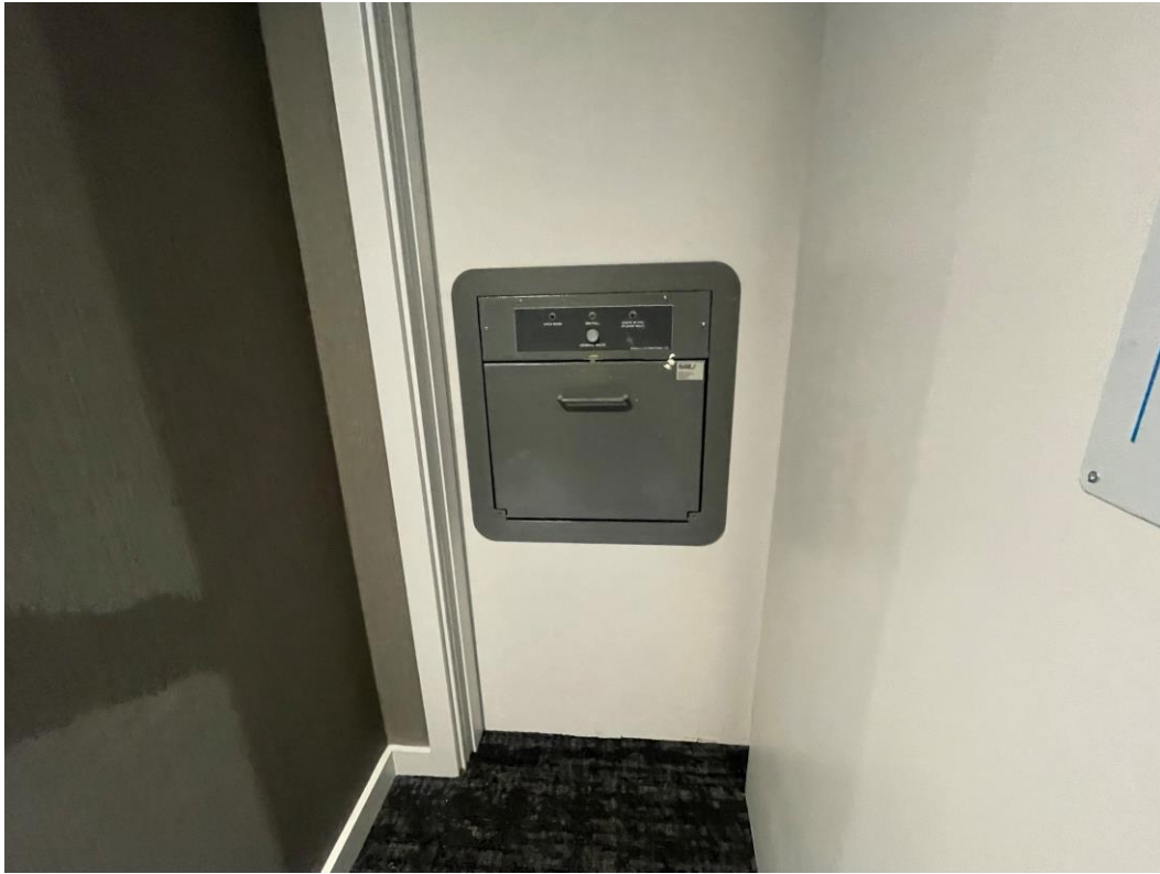
Bin chute installed
