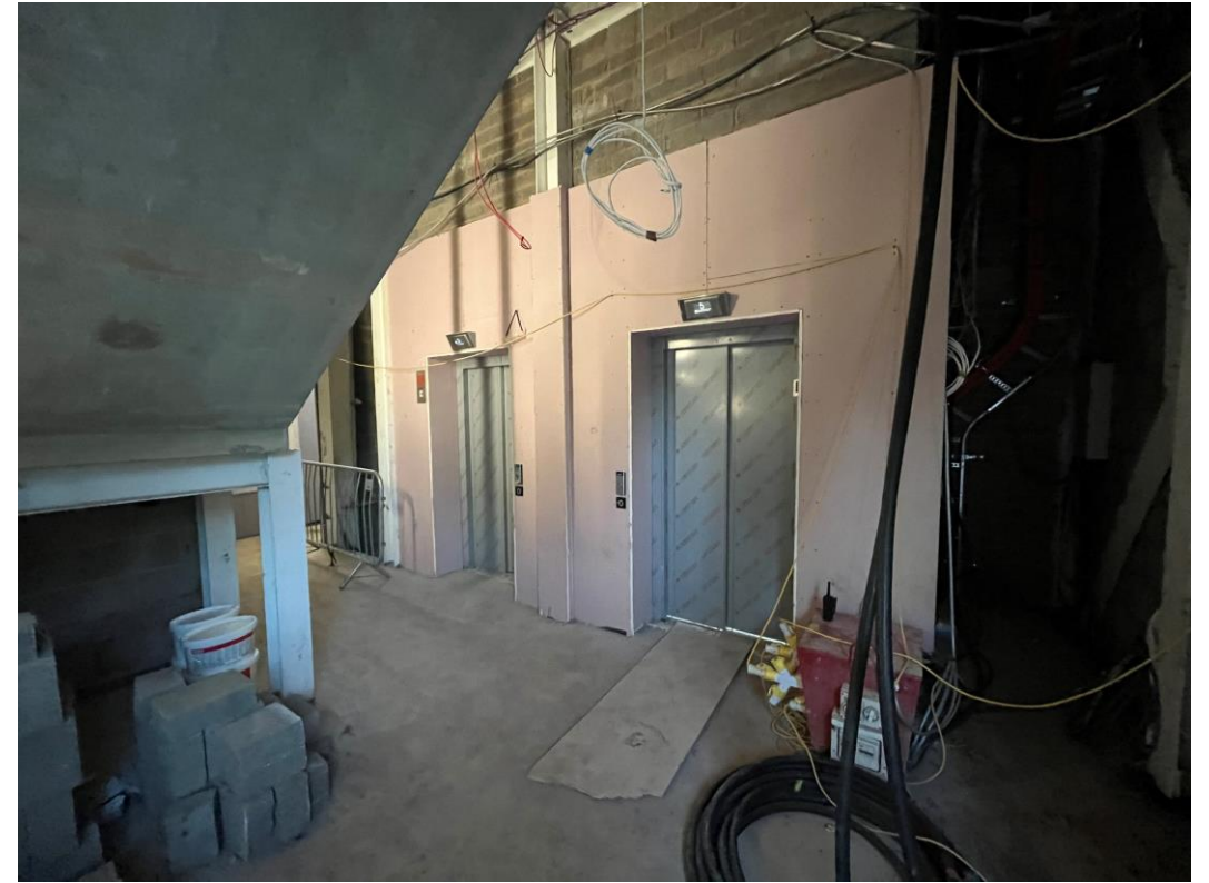
Ground Floor lift area
