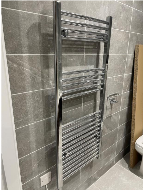
Towel radiator installed
