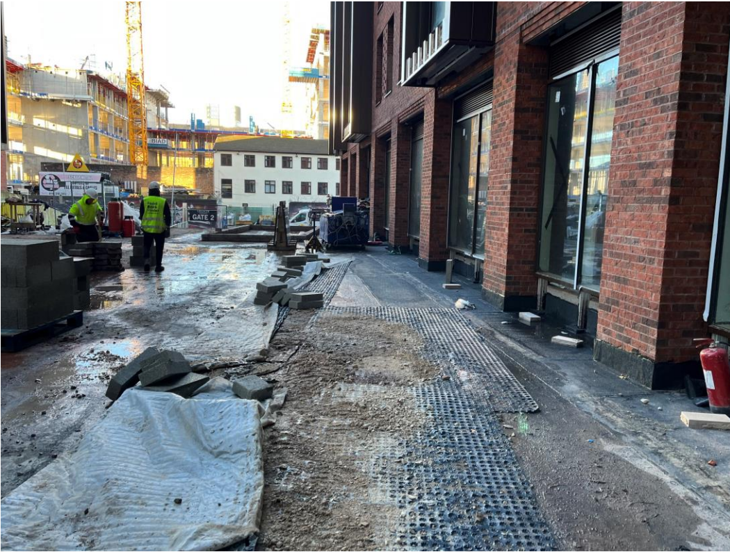
Deck drain installed
