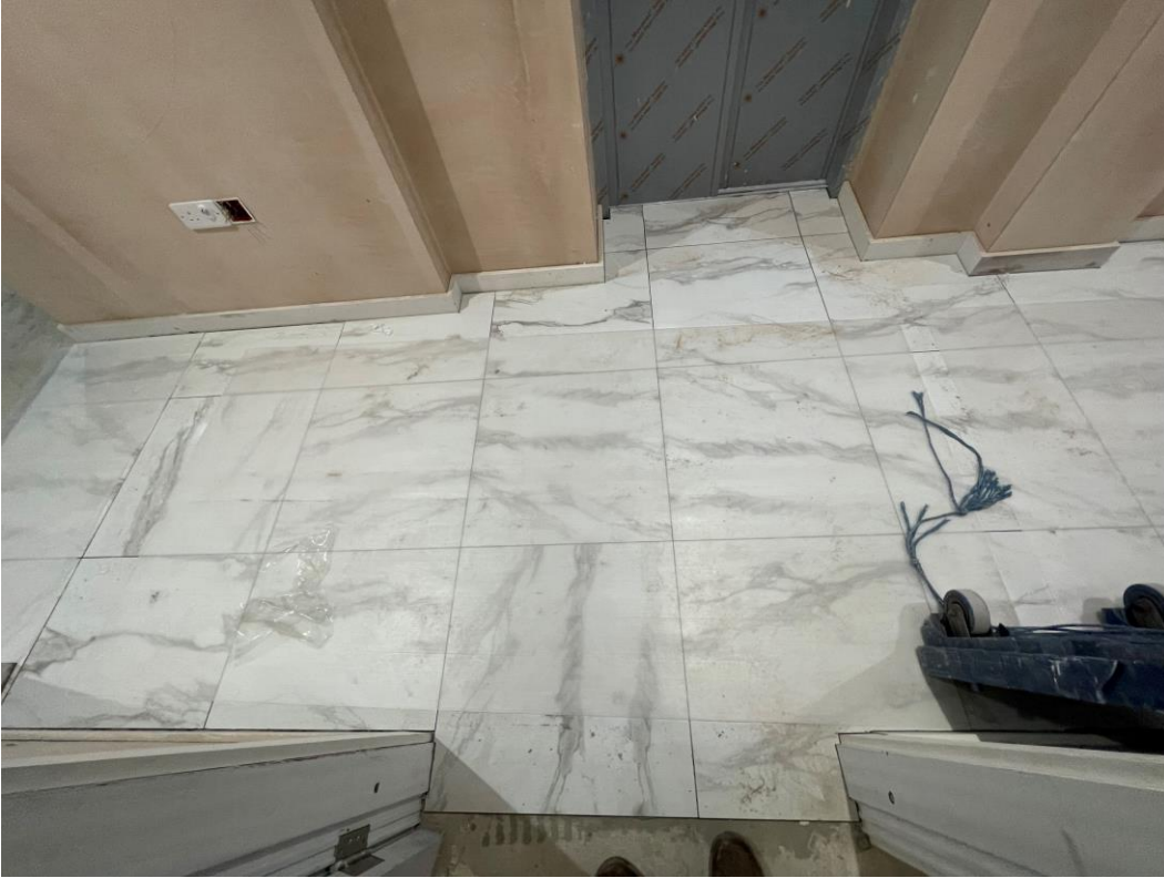
Lift area floors tiled
