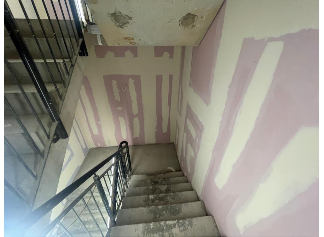
Tape & jointing commenced to stairwell areas
