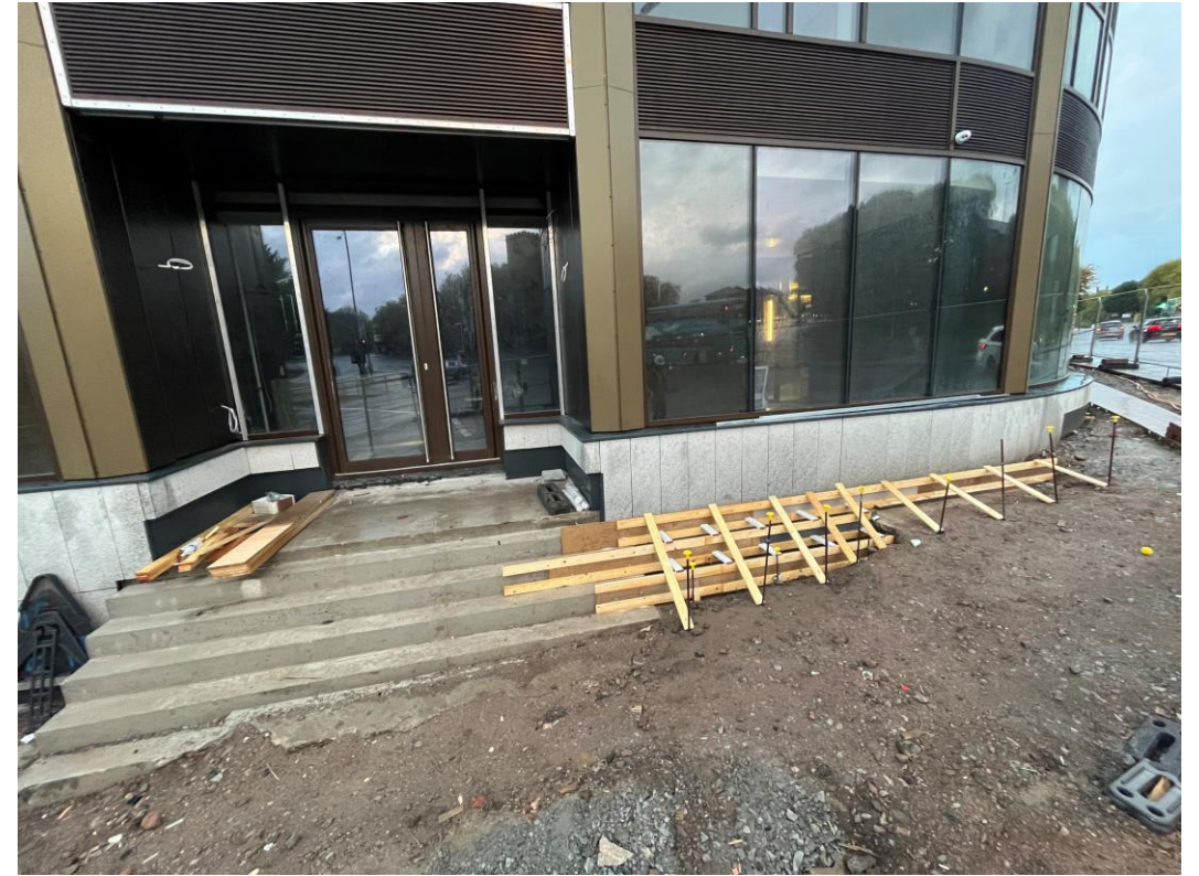
External step formwork in place
