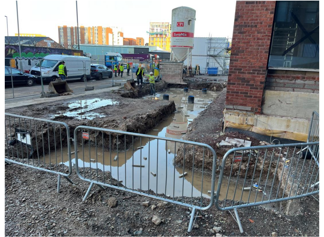
Preparations ongoing for strip foundation concrete pour external staircase and ramp
