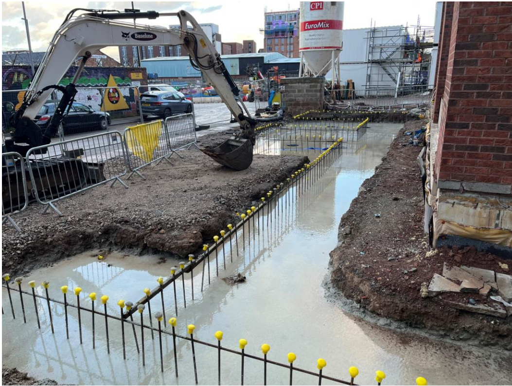
Strip foundations poured for external staircase and ramp
