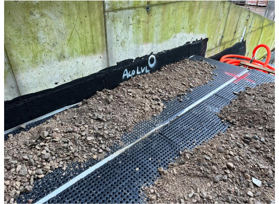
Deck drain installed
