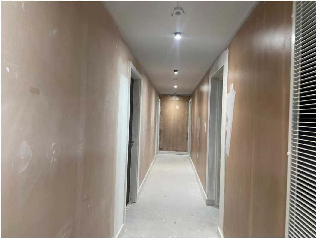
Circulation area finishes
