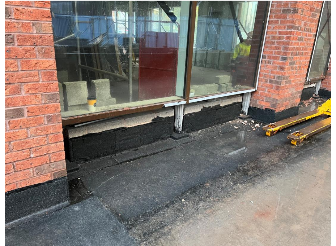
Bitumen Felt upstand from podium to Block B
