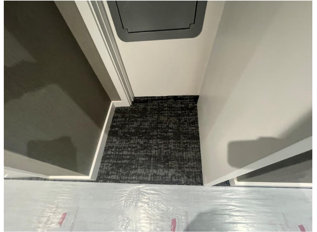
Corridor carpets installed
