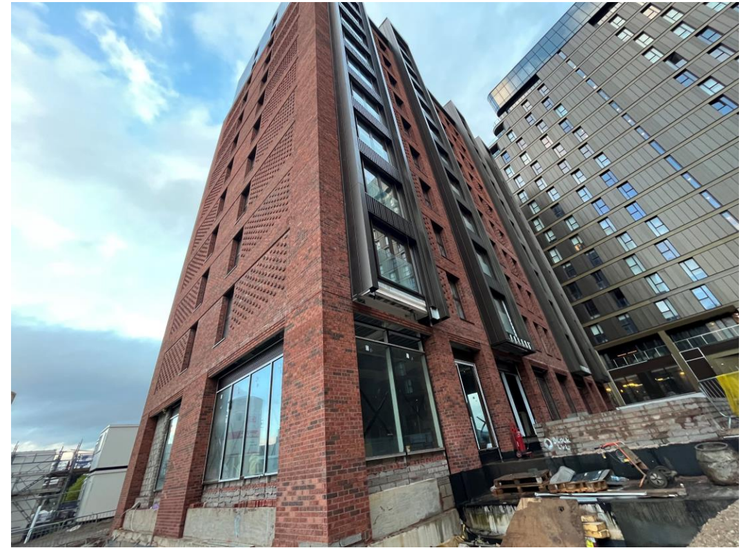
Brickwork façade nearing completion
