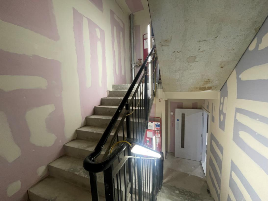
Tape & jointing commenced to stairwell areas
