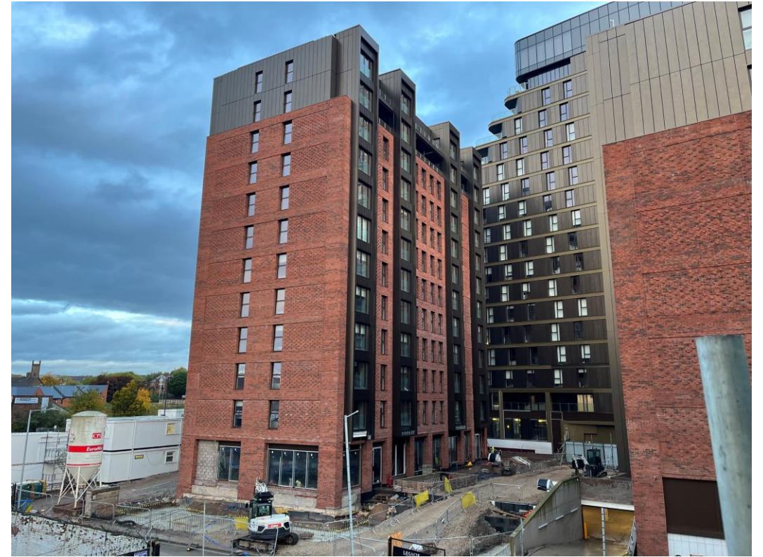
Block B – Viewed from Block D
