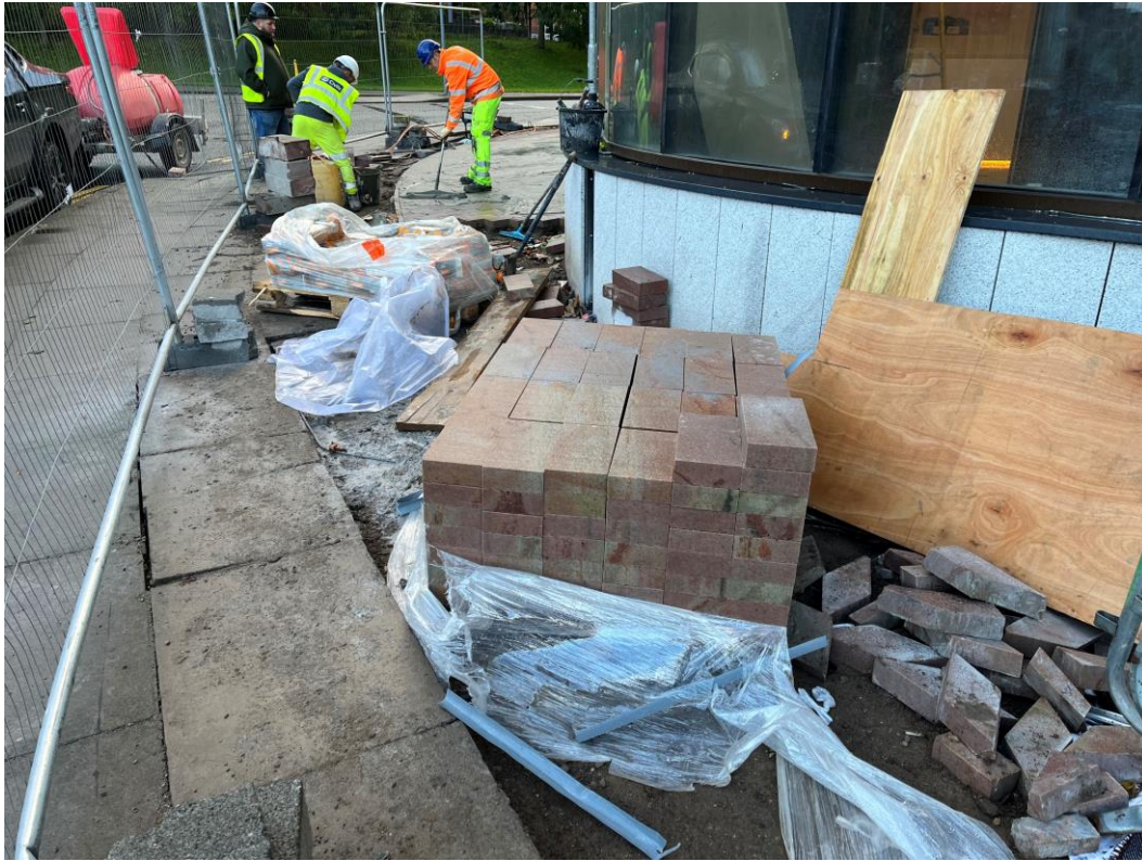
Paving flags onsite for installation
