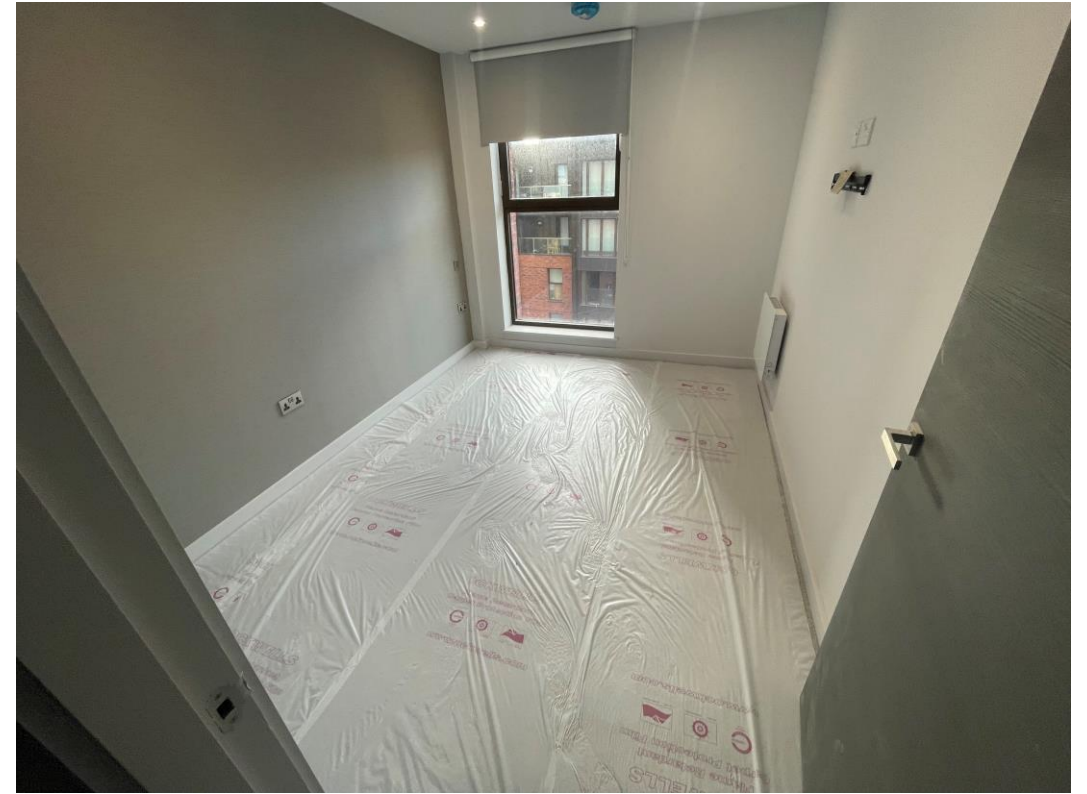
Carpets installed & protected
