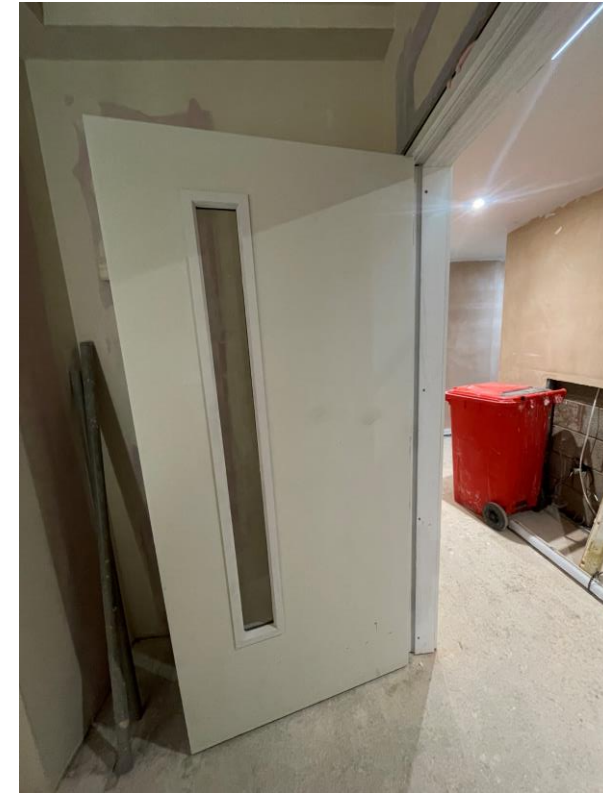
Circulation doors installed
