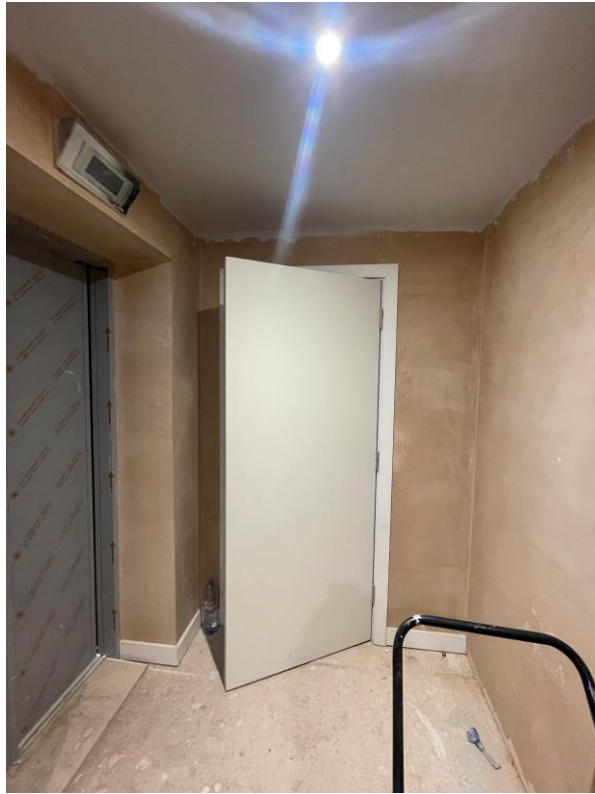
Electric meter cupboard door installed
