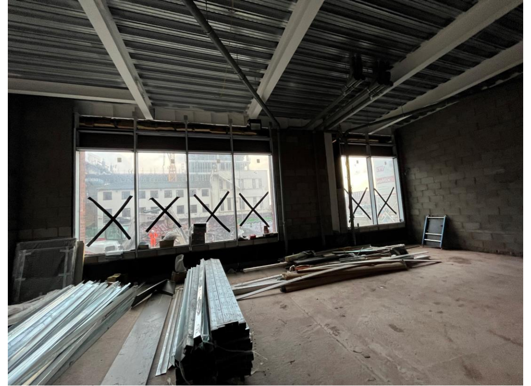
Curtain wall installed
