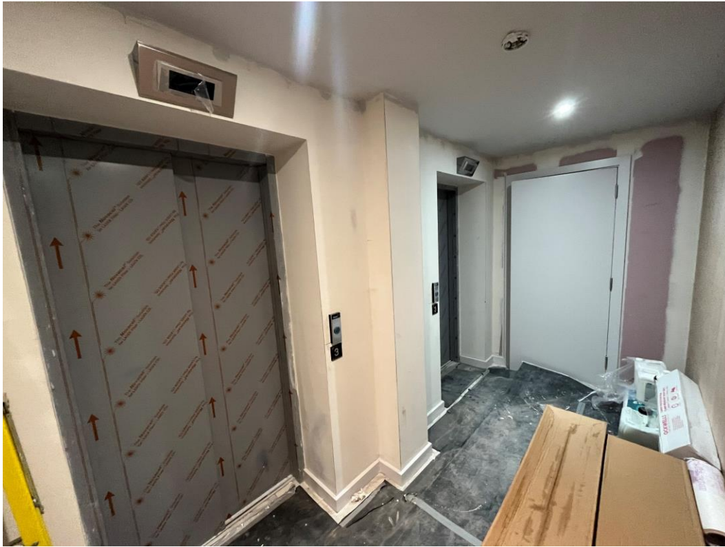
Lift area finishes
