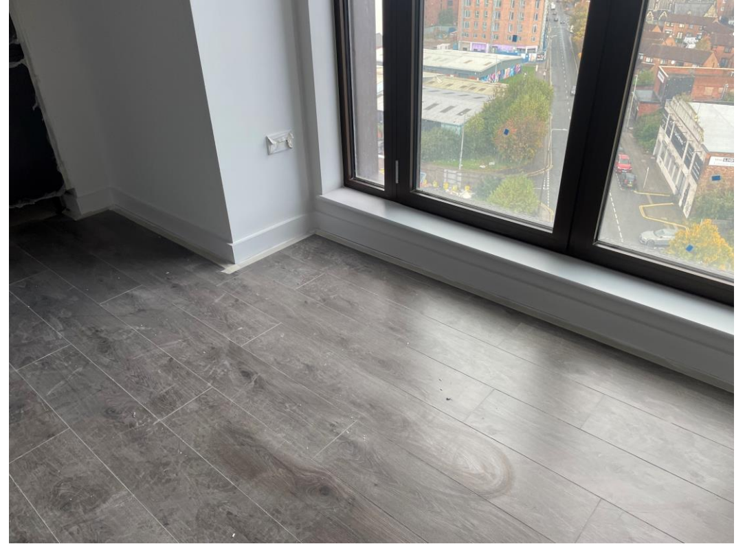
2 nd Fix joinery decoration ongoing
