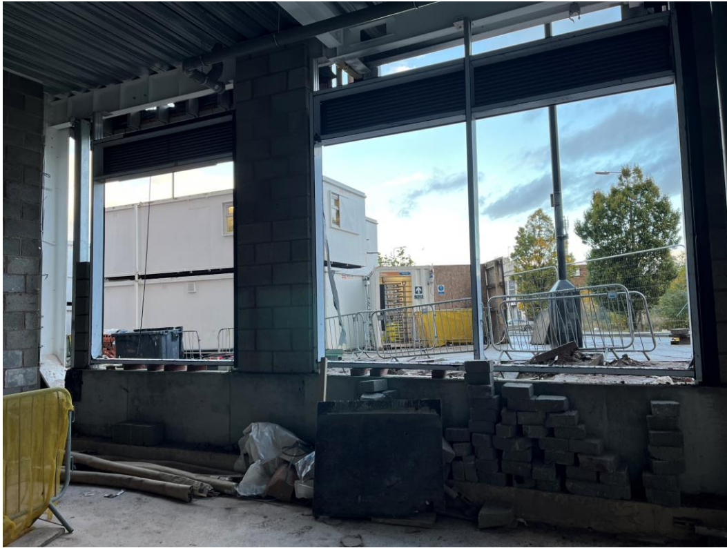
Curtain wall installation ongoing
