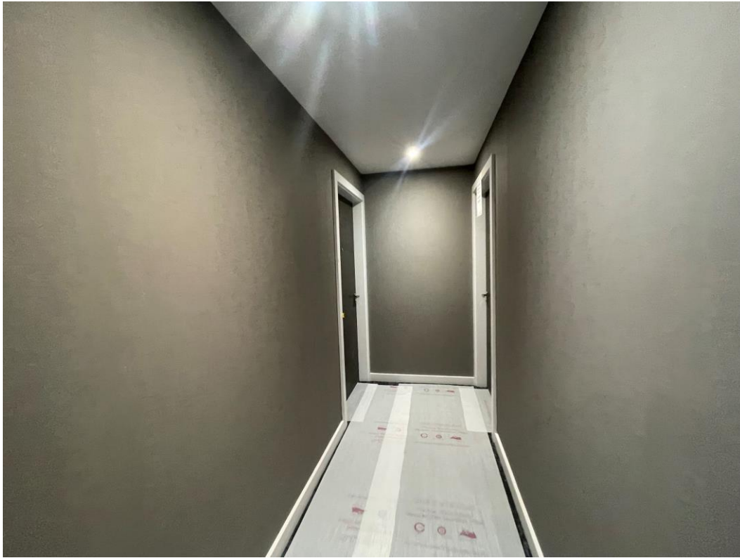
Wallpaper installed to circulation areas
