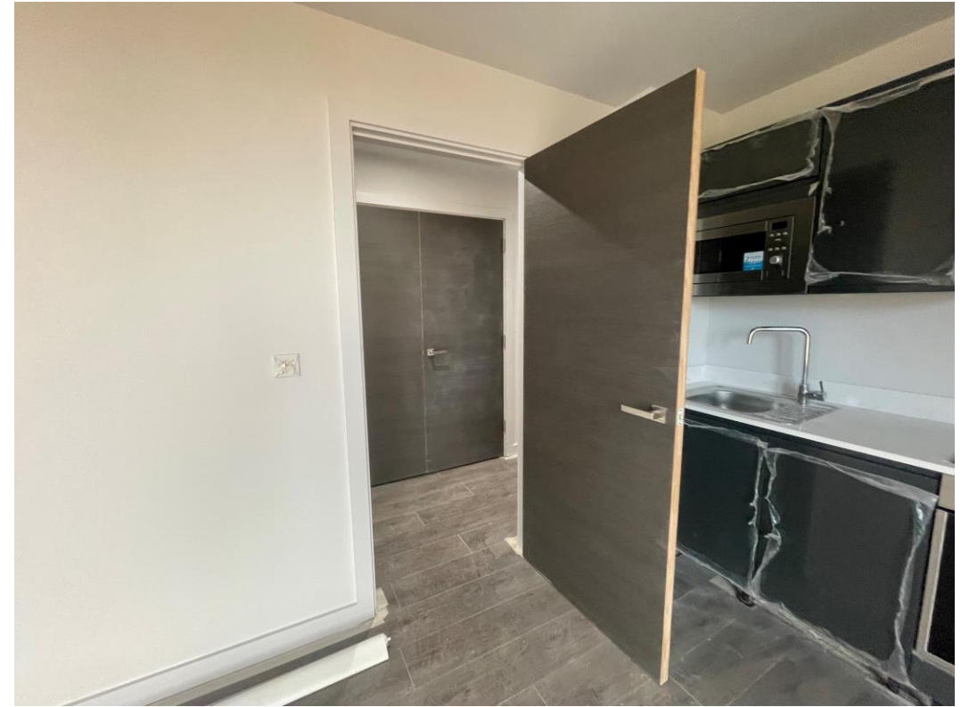
Doors & ironmongery installed
