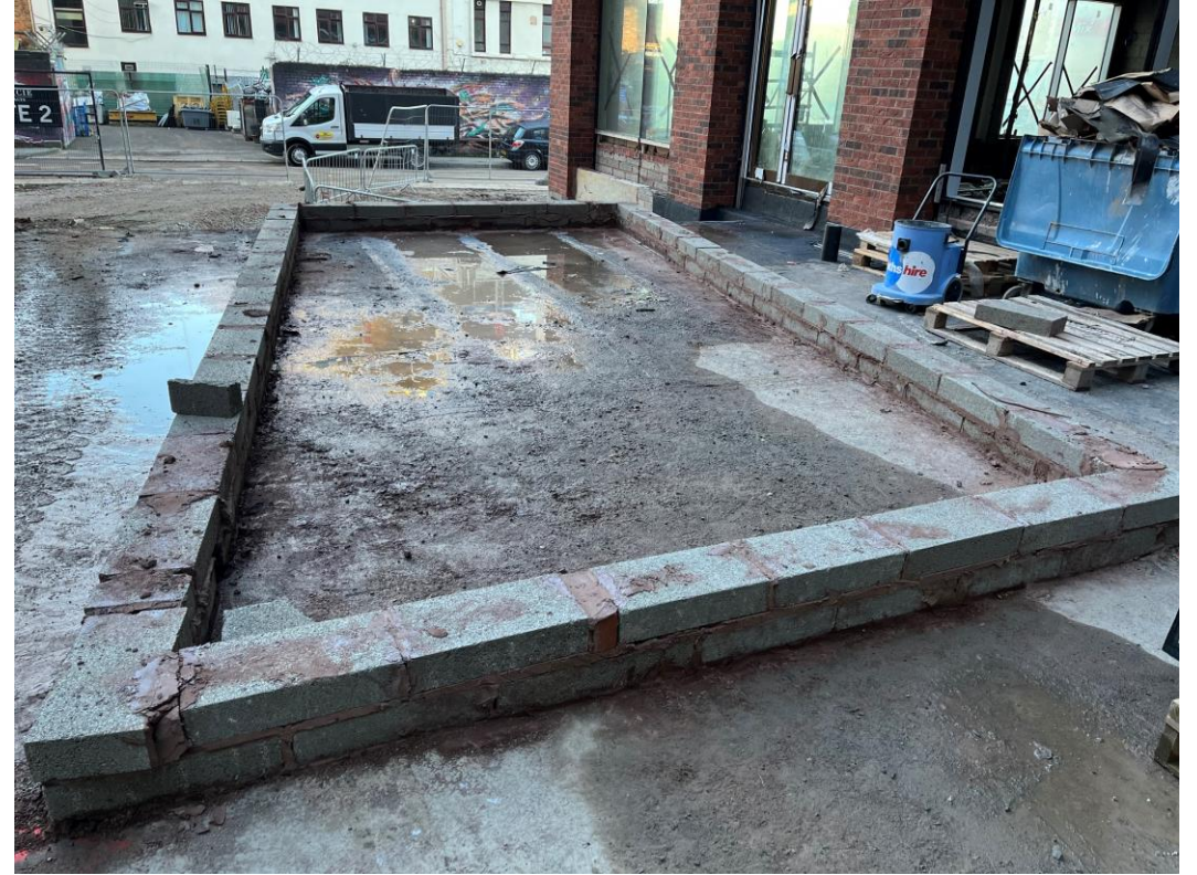
Raised planter construction ongoing
