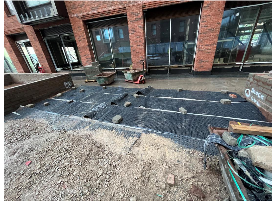
Deck drain installed
