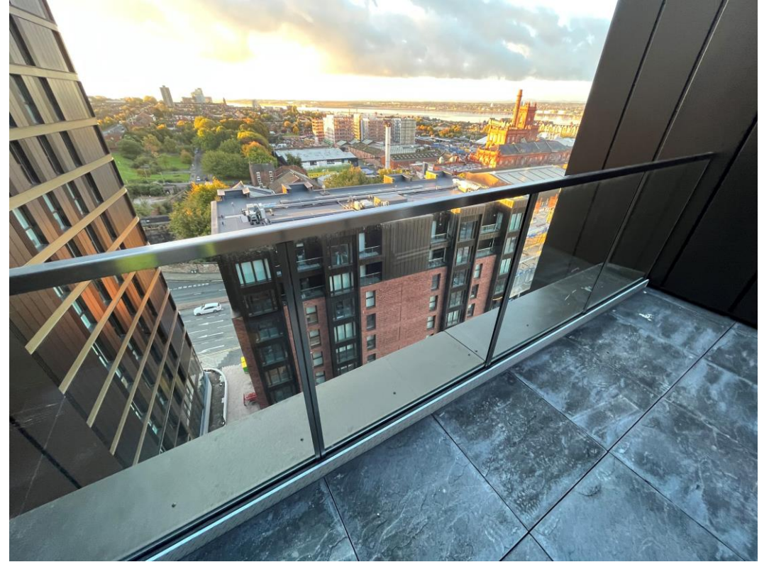
Glazed balustrade installed
