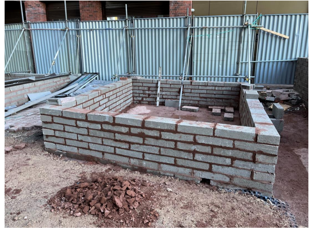
Raised planter construction ongoing
