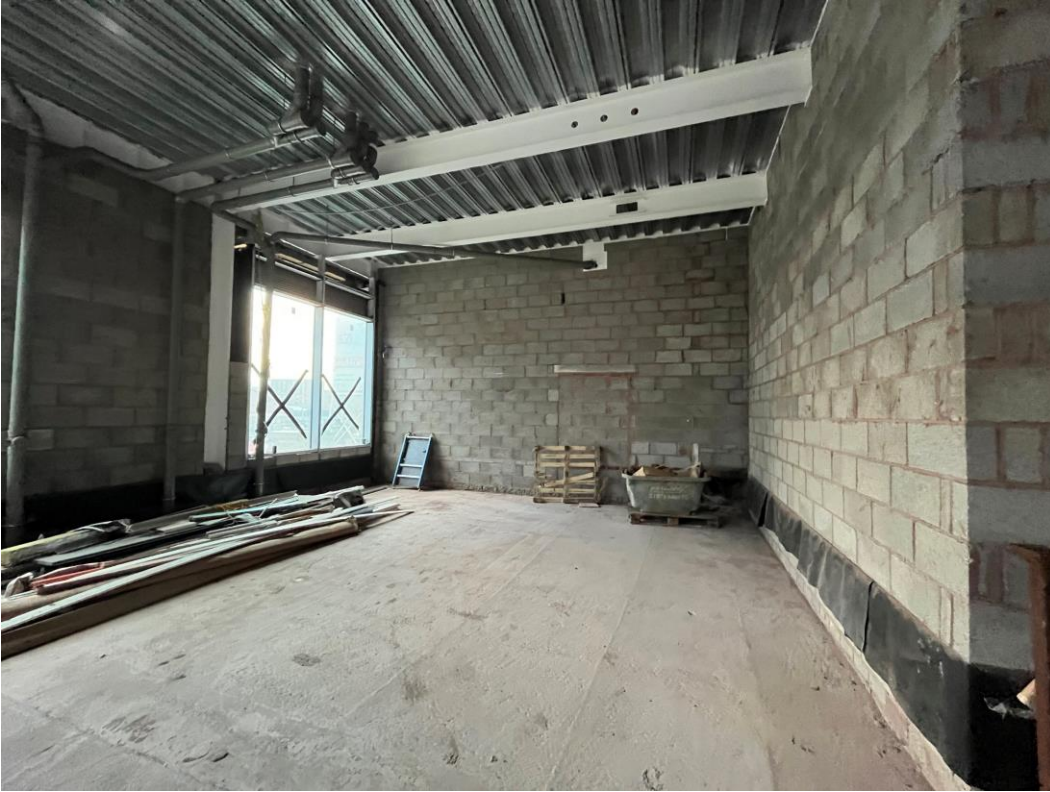
Commercial unit under construction
