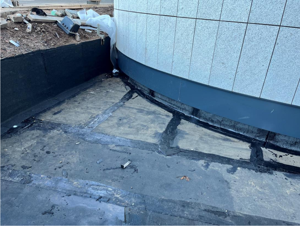
Waterproof membrane in place to ramp to St George Street
