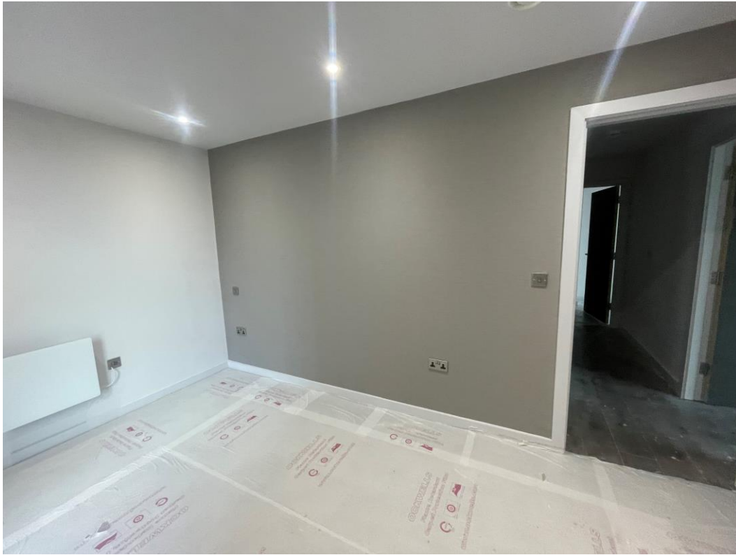
Bedroom wallpaper installed
