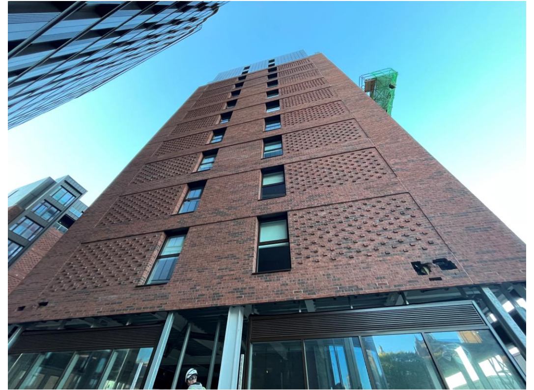
Brickwork façade nearing completion
