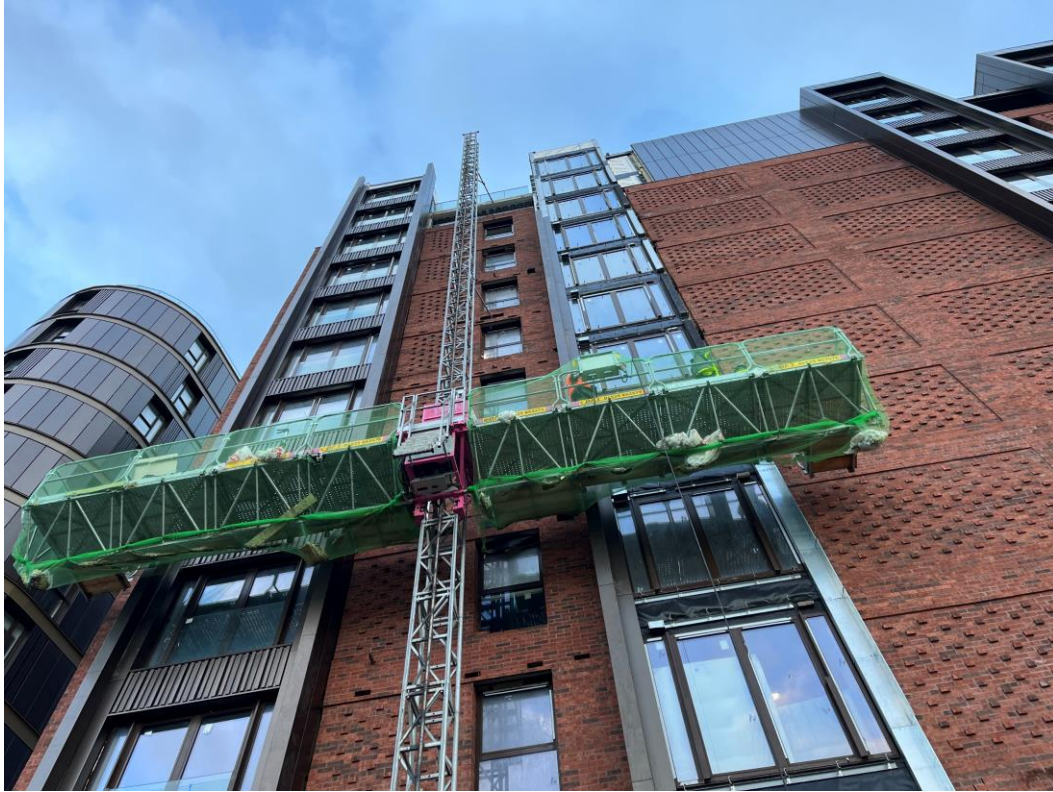
Cladding installation nearing completion
