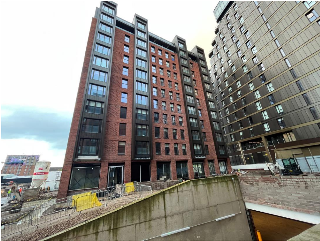
Brickwork façade nearing completion
