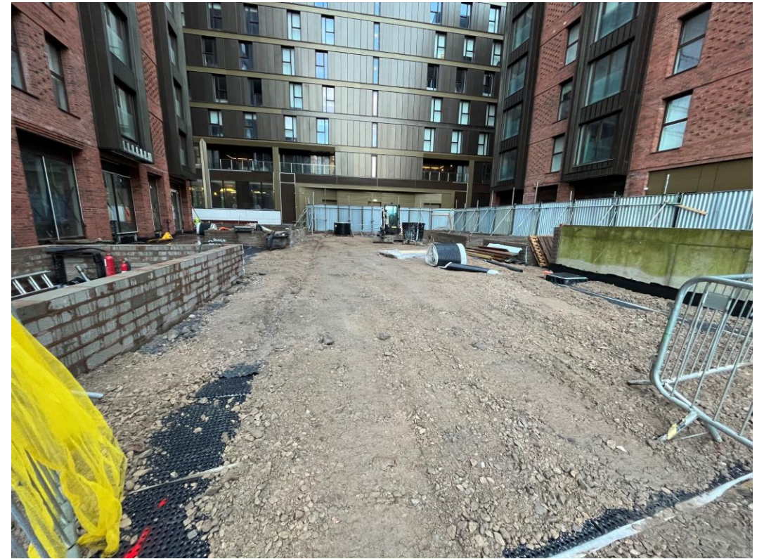
Podium build up
